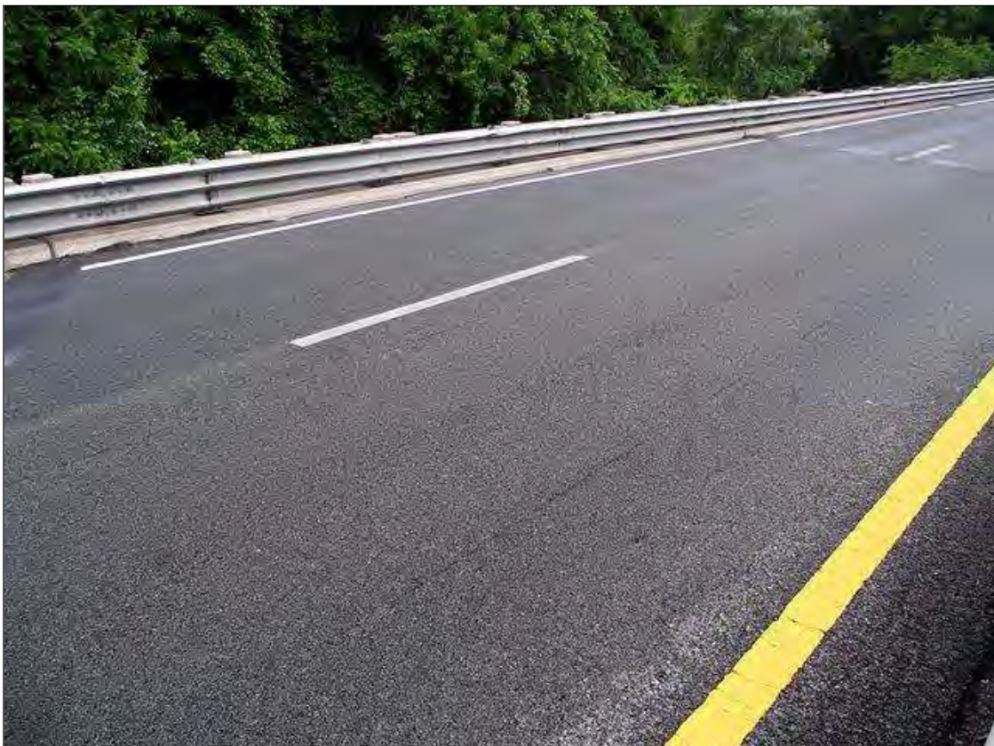
SPAN 2 OVERVIEW - ALL SPANS SIMILAR
