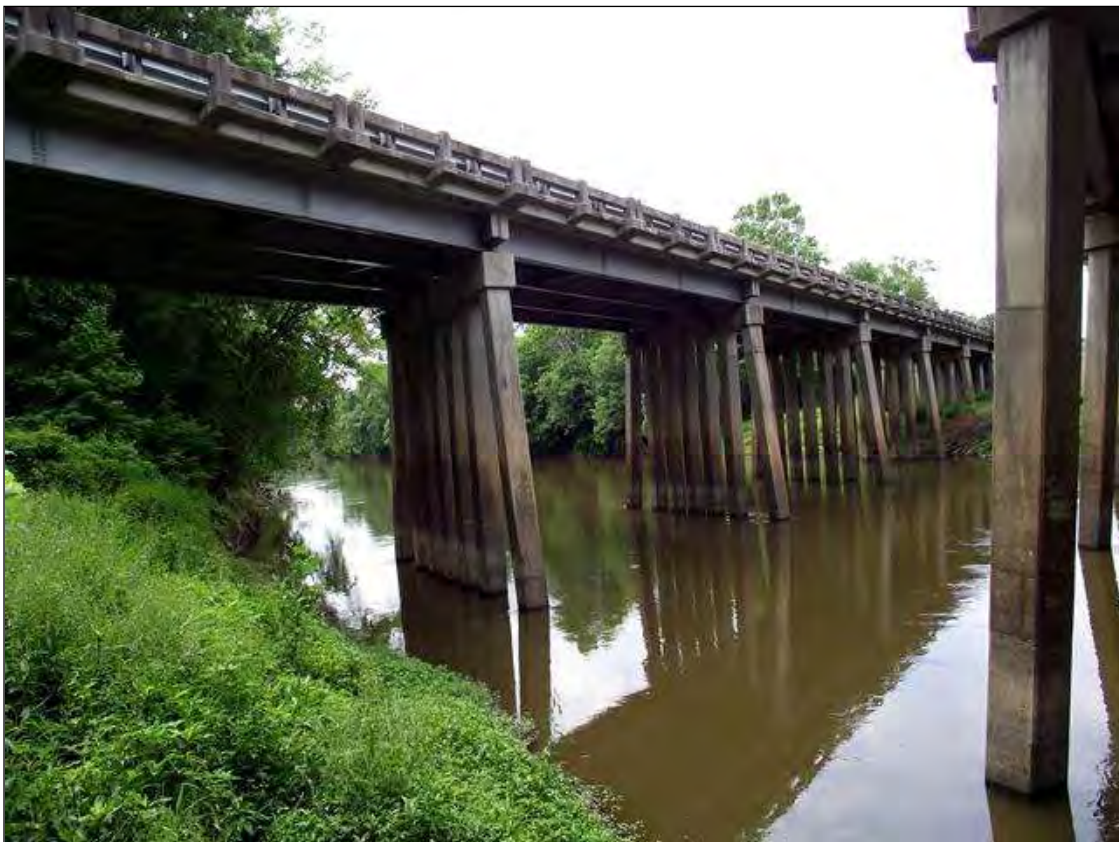
LOOKING EAST DOWNSTREAM TOWARDS THE NORTHBOUND STRUCTURE
