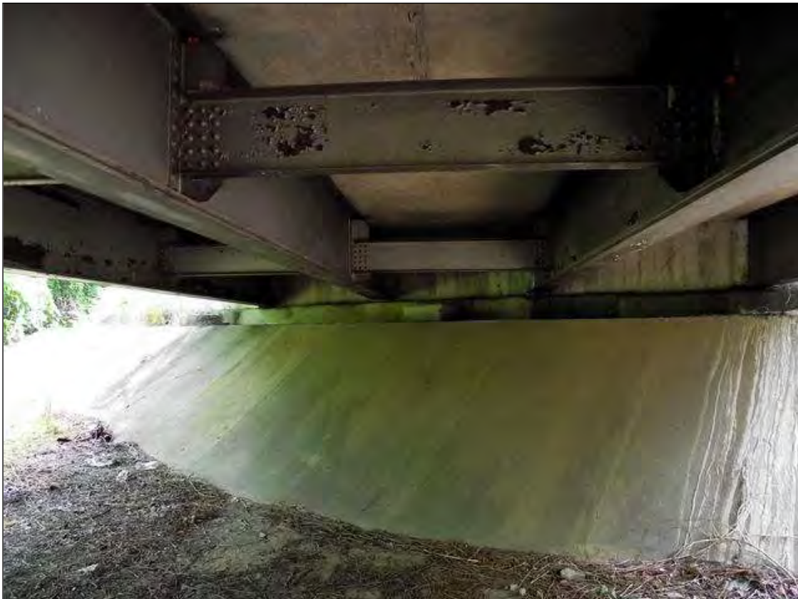
END BENT 2 OVERVIEW
