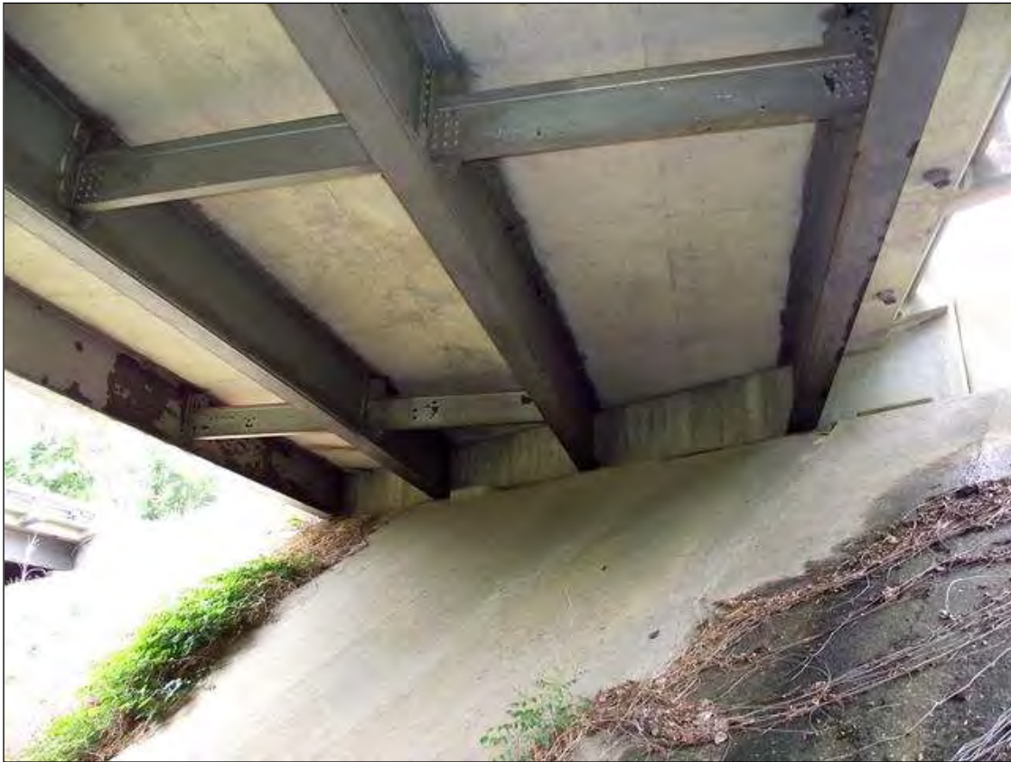
END BENT 1 OVERVIEW
