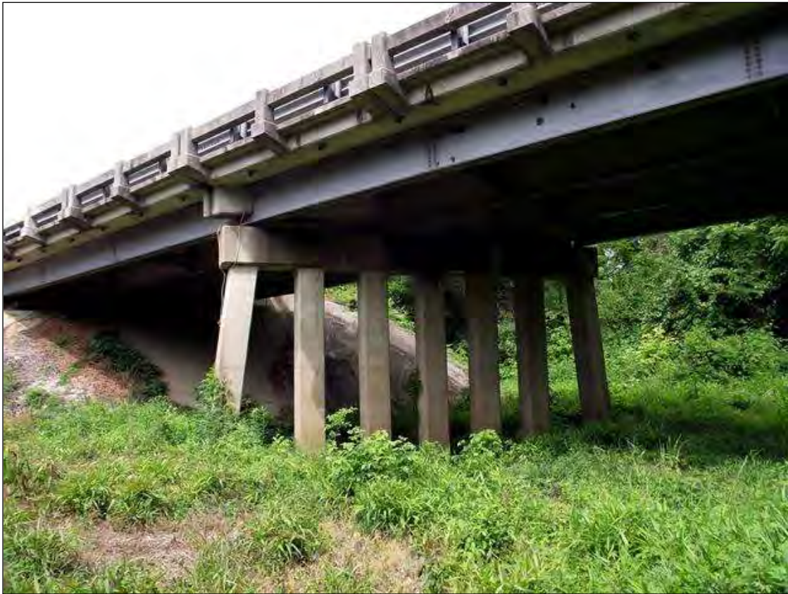
BENT 1 SPAN 2 SIDE - ALL BENTS SIMILAR
