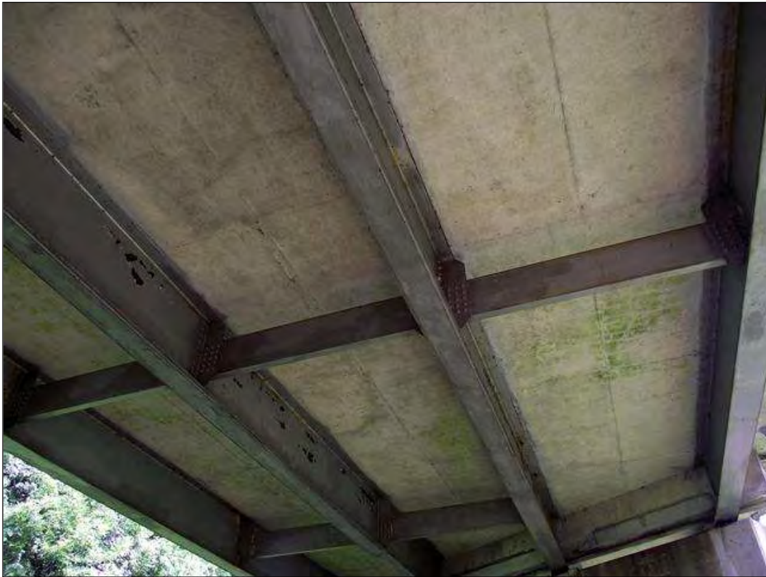
SUPERSTRUCTURE OVERVIEW - ALL SPANS SIMILAR
