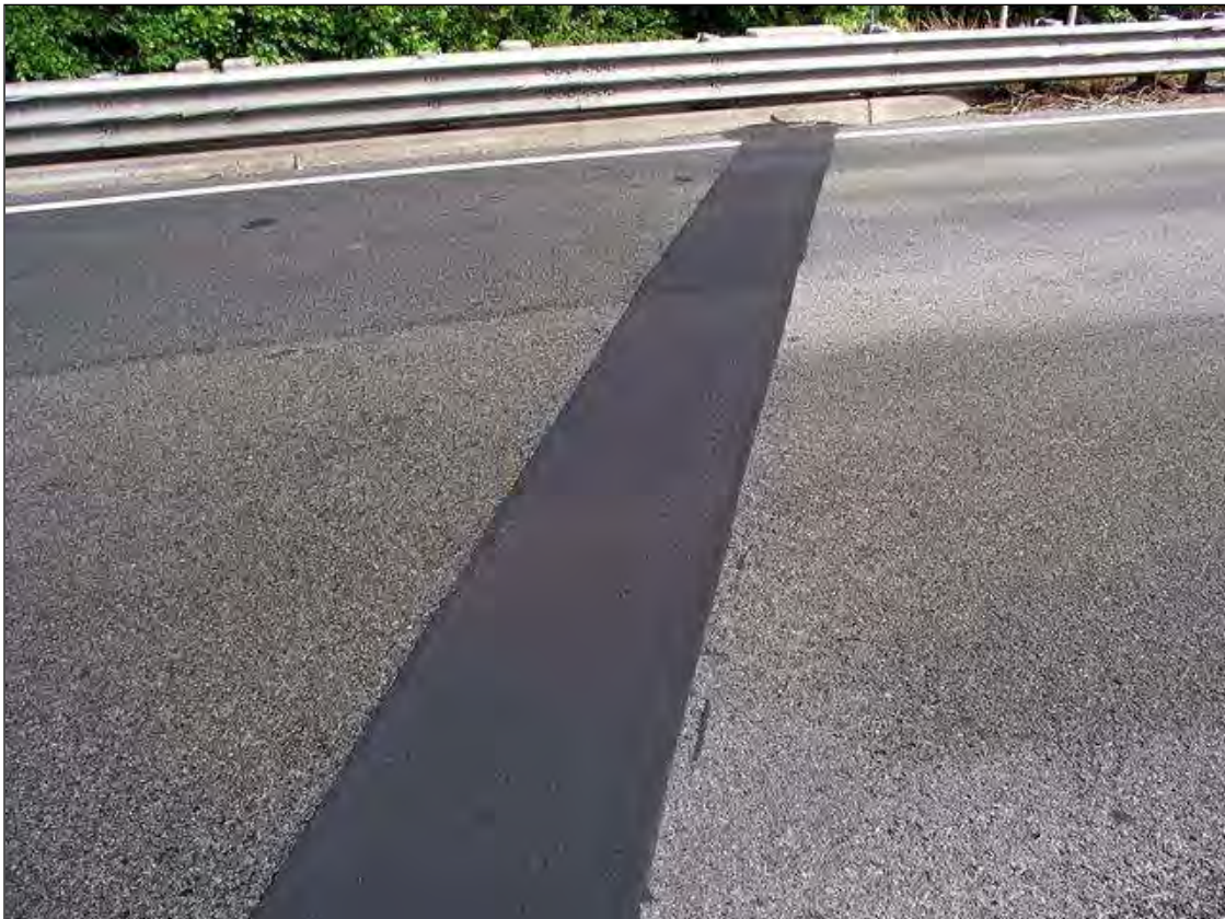
JOINT AT END BENT 2
