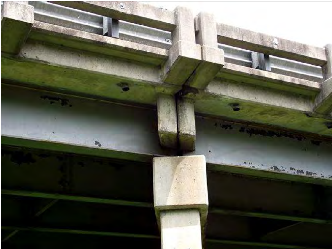
SUPERSTRUCTURE OVER END OF CAP
