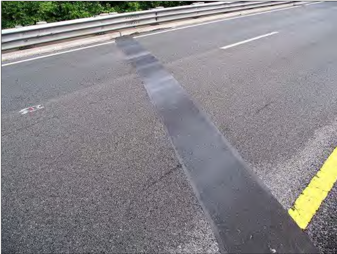
JOINT AT BENT 1 - ALL OTHER BENT JOINTS SIMILAR
