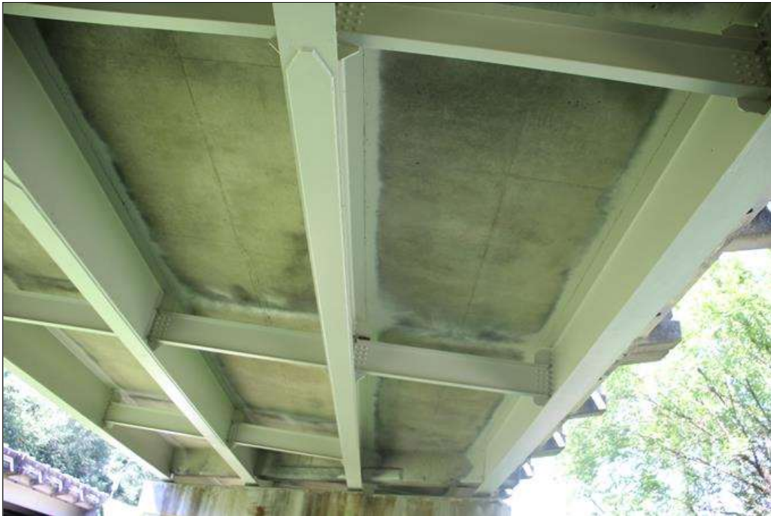
SUPERSTRUCTURE UNDERSIDE SPAN 2. NOTE NEW PAINT.
