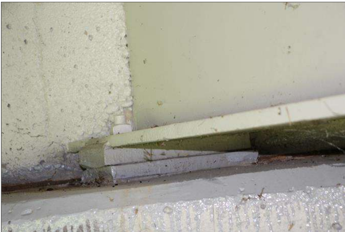
BEARING AT END BENT 2 BEAM 2. NOTE NEW PAINT.
