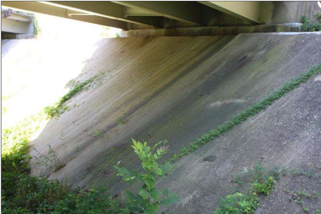
SLOPE PROTECTION AT END BENT 1
