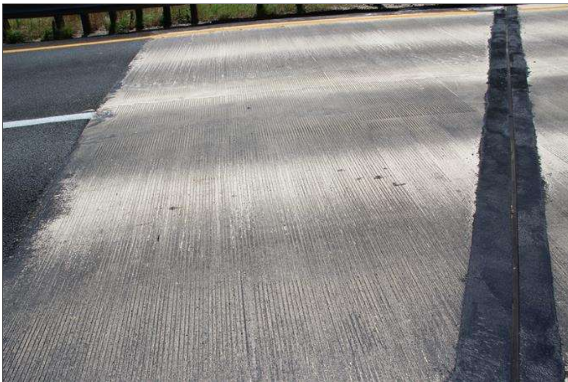
NORTH APPROACH SLAB
