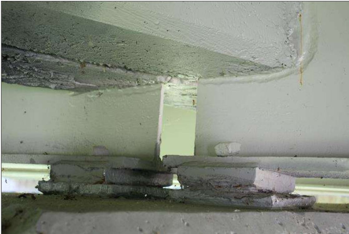
BEARINGS AT BENT 1 BEAM 2
