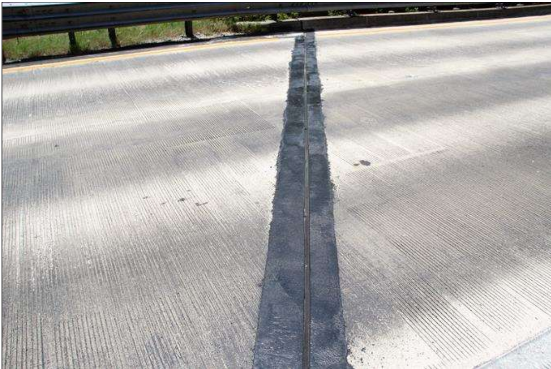
DECK JOINT AT END BENT 2. TYPICAL AT END BENT 1.
