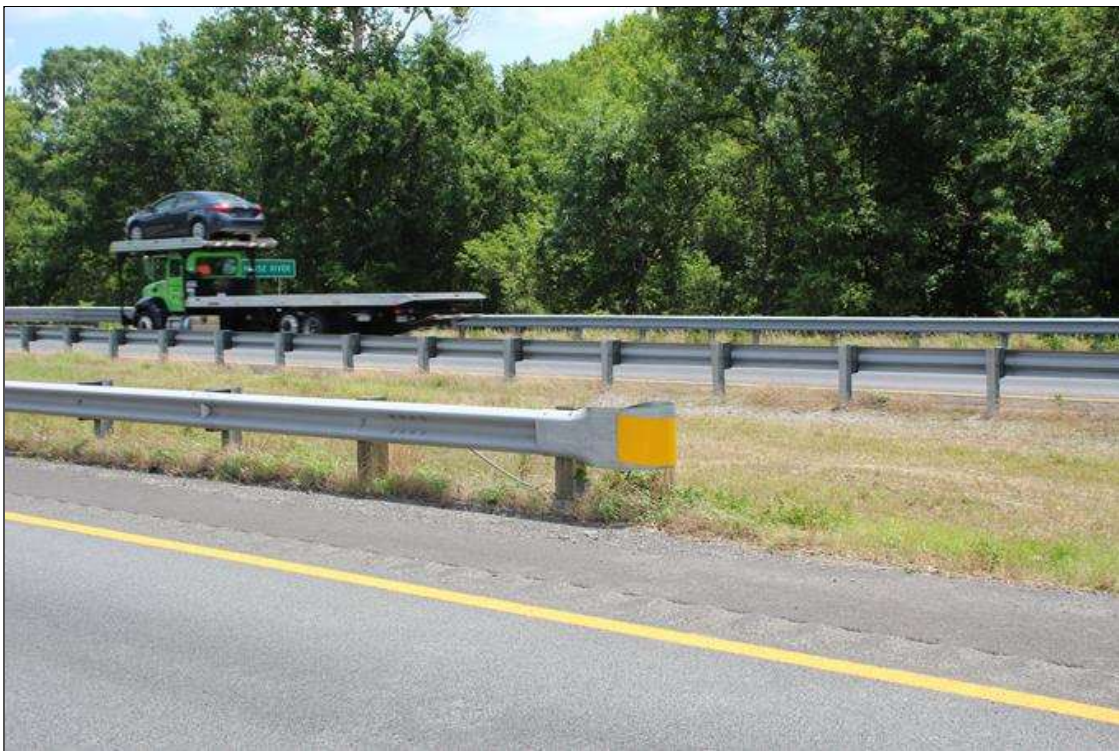
GUARDRAIL END TERMINAL AT SOUTHEAST CORNER
