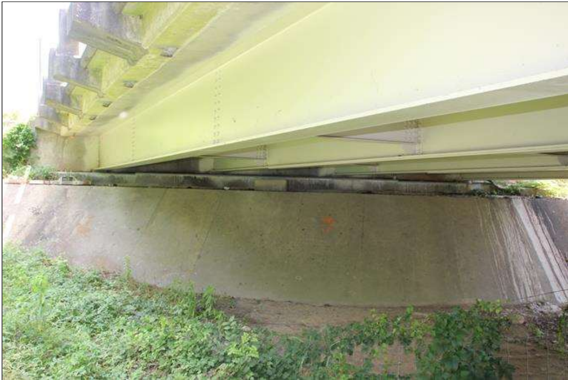
SLOPE PROTECTION AT END BENT 2
