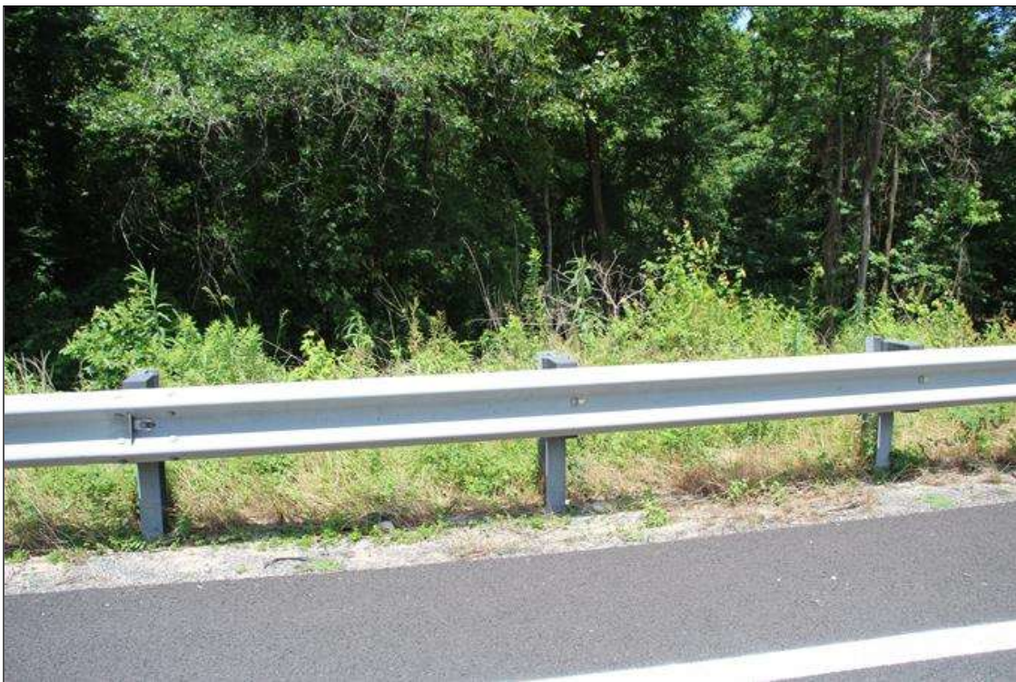
POST SPACING MID LENGTH NORTHWEST CORNER
