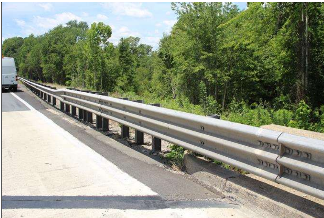
POST SPACING AT BRIDGE SOUTHWEST CORNER
