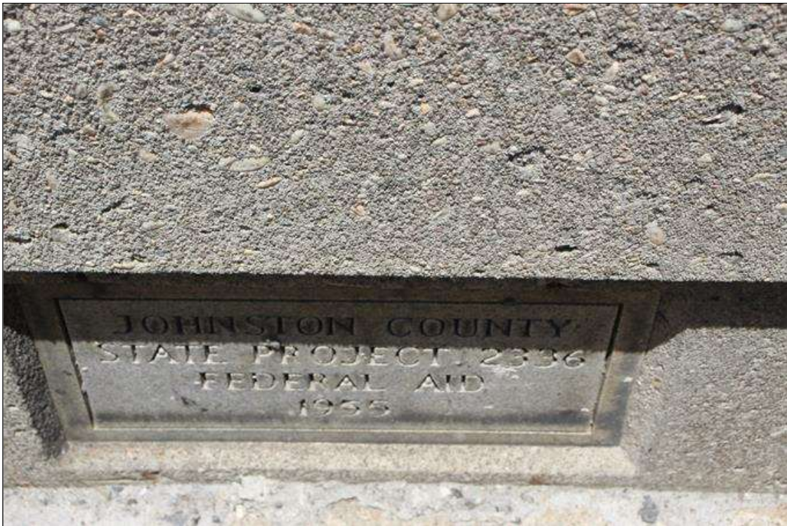
BRIDGE PLAQUE AT NORTHWEST CORNER. TYPICAL AT SOUTHEAST CORNER.
