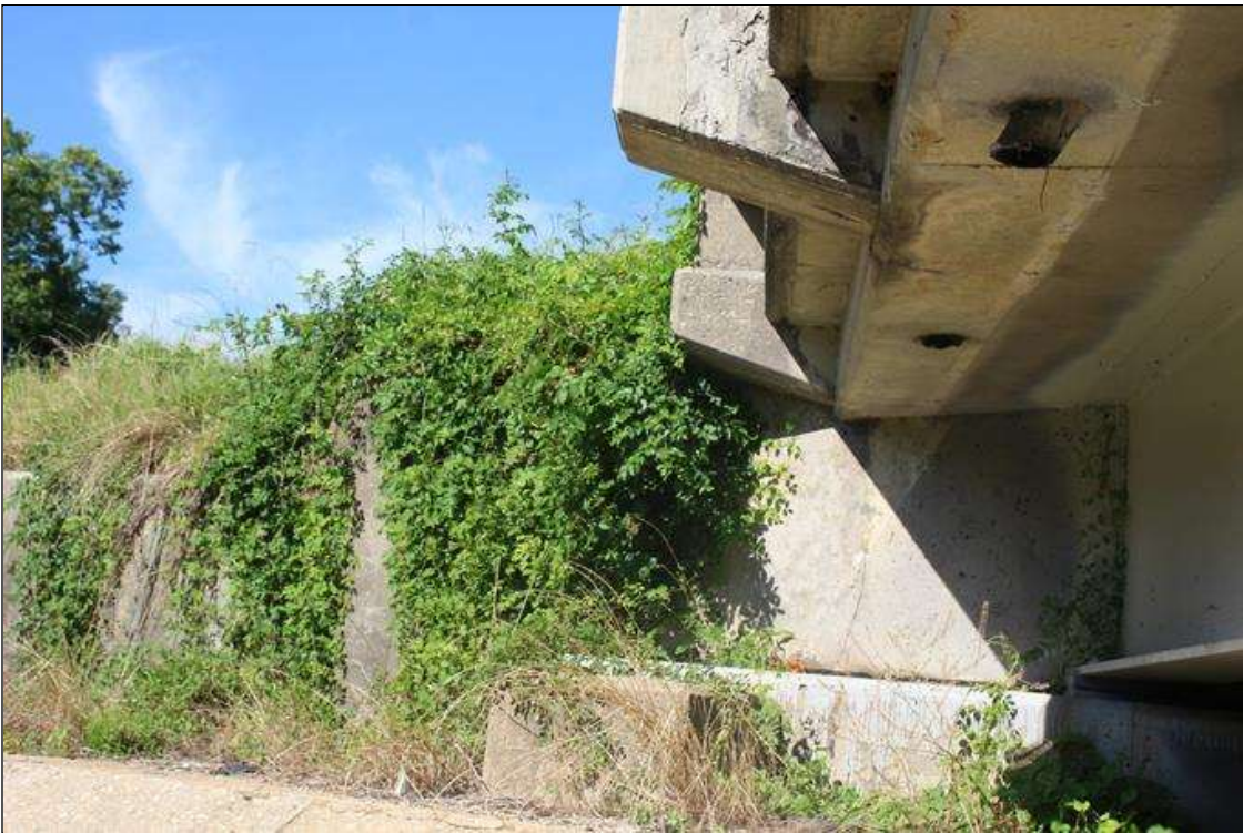
SOUTHEAST WINGWALL. NOTE HEAVY VEGETATION.
