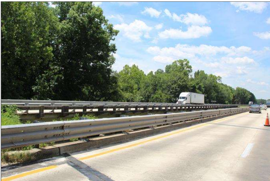
RIGHT BRIDGE RAIL
