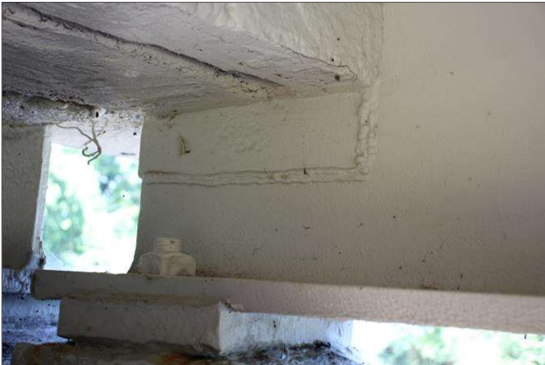
WELDED REPAIR TO WEB BELOW END DIAPHRAGM, AT BENT 5.
