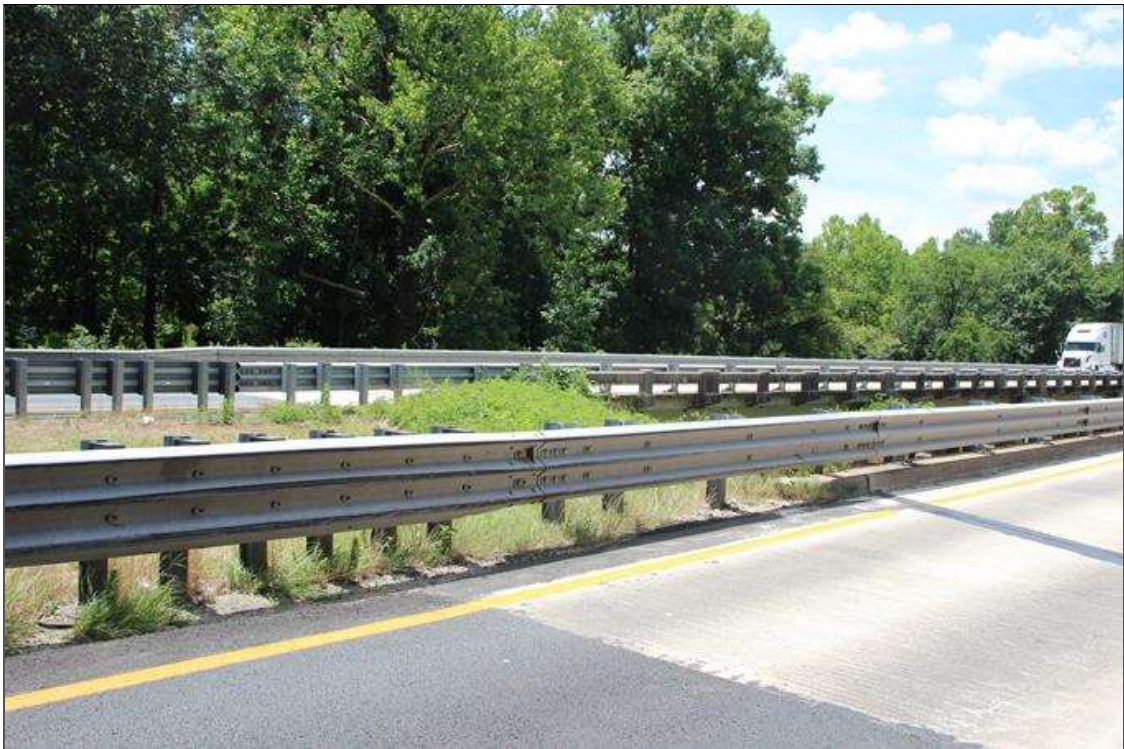
POST SPACING AT BRIDGE NORTHEAST CORNER
