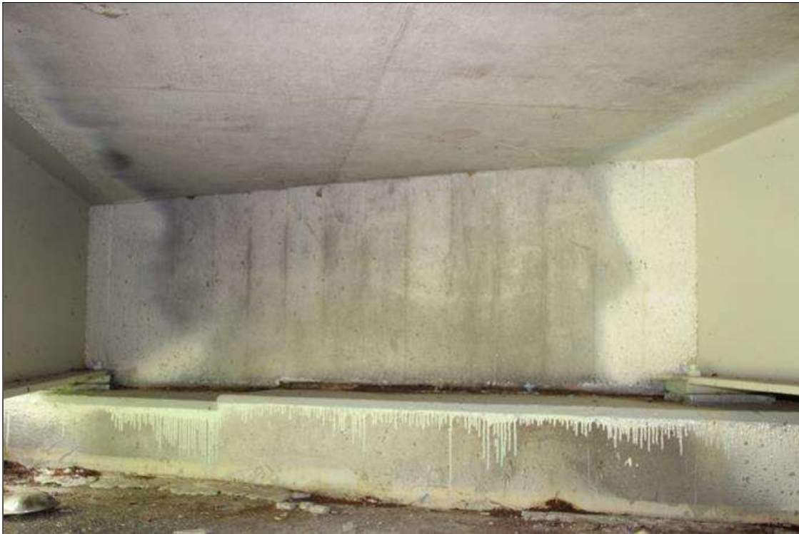
BACKWALL AND CAP AT END BENT 2 BAY 1
