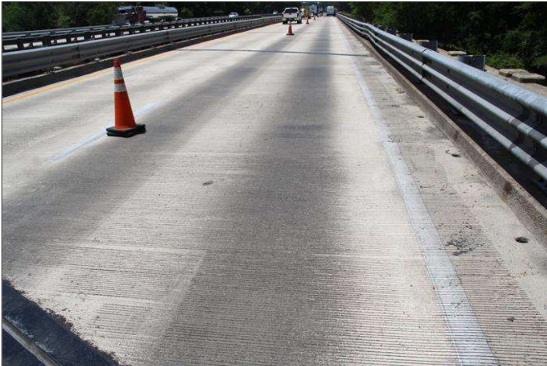
TOP OF DECK. NEW LMC OVERLAY SINCE PREVIOUS INSPECTION.
