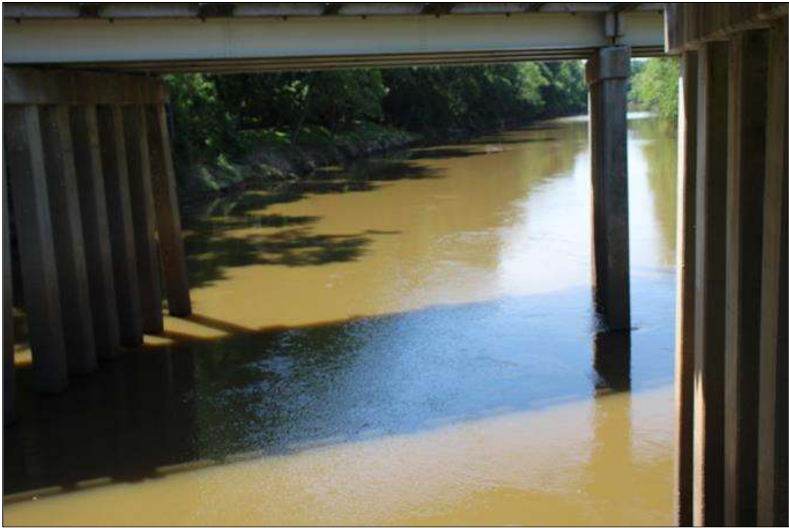
DOWNSTREAM FROM UNDER THE BRIDGE
