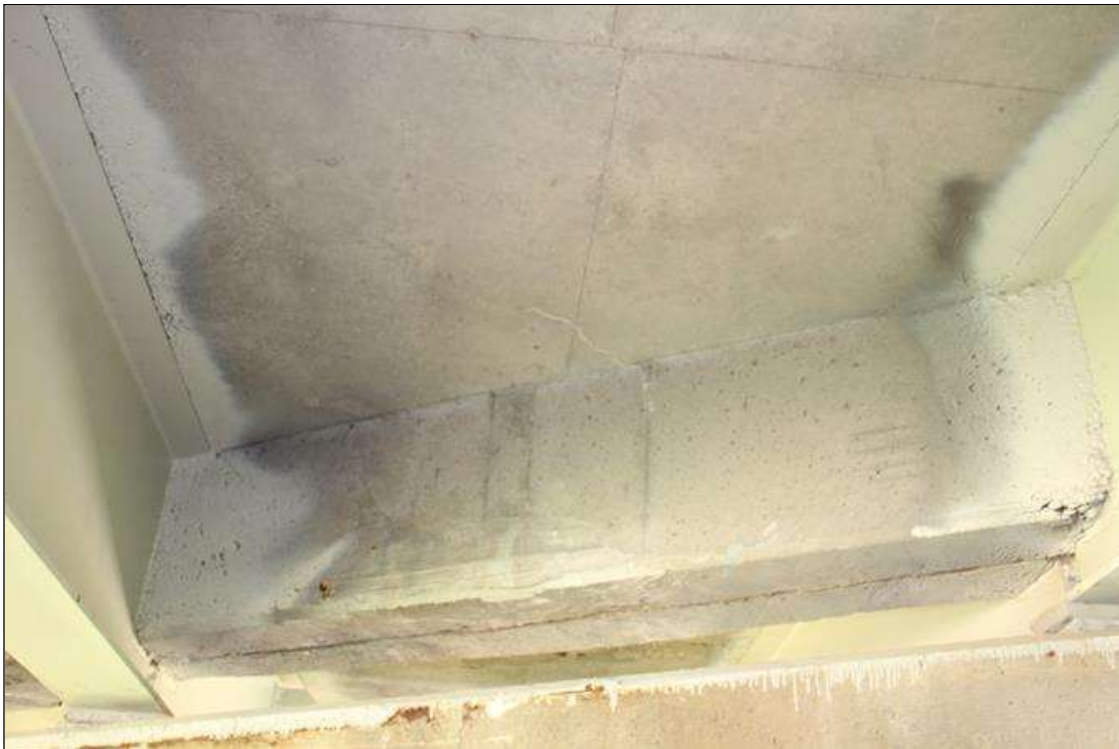
END DIAPHRAGM AT BENT 7 BAY 2
