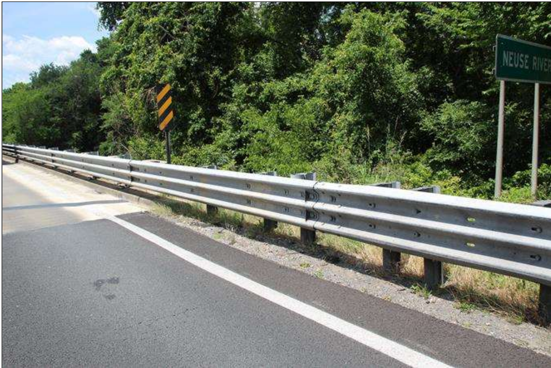
POST SPACING AT BRIDGE NORTHWEST CORNER
