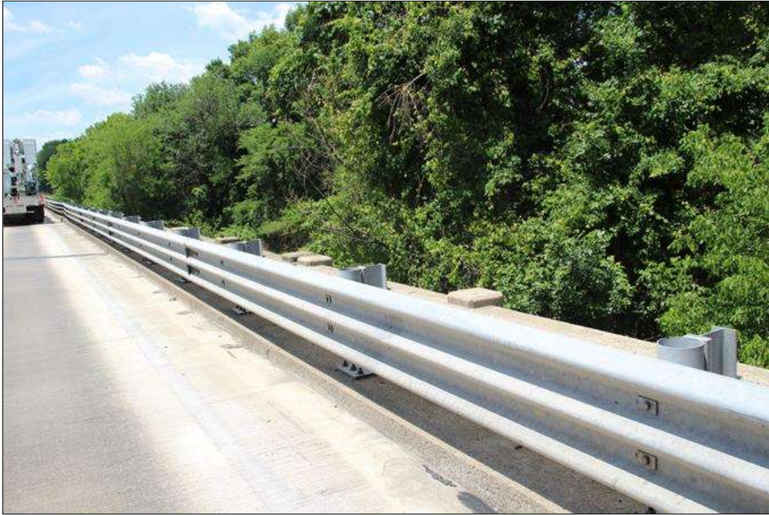
LEFT BRIDGE RAIL
