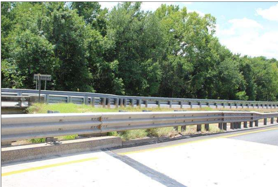
POST SPACING AT BRIDGE SOUTHEAST CORNER
