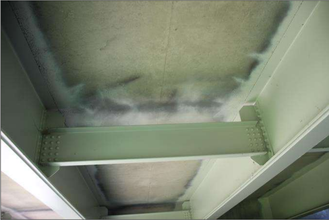
INTERMEDIATE DIAPHRAGM IN SPAN 1 BAY 2
