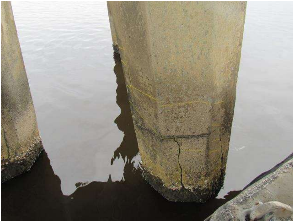
Bent 37 Saved Pile 4: 42" X 36" DELAMINATION ON NORTH AND WEST FACE, 7' FROM BOTTOM OF CAP
