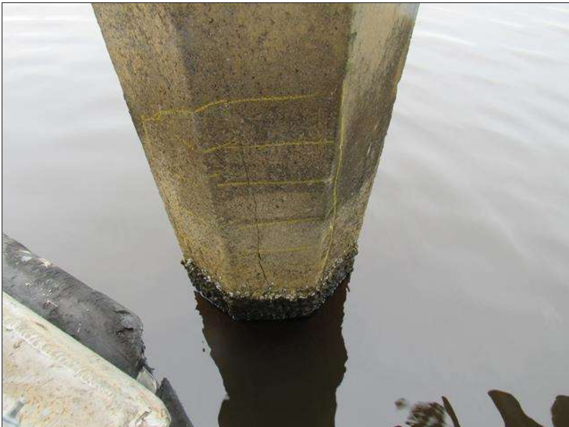
Bent 37 Saved Pile 1: 32" X 19" DELAMINATION ON SOUTH FACE LOCATED 8' FROM BOTTOM OF CAP
