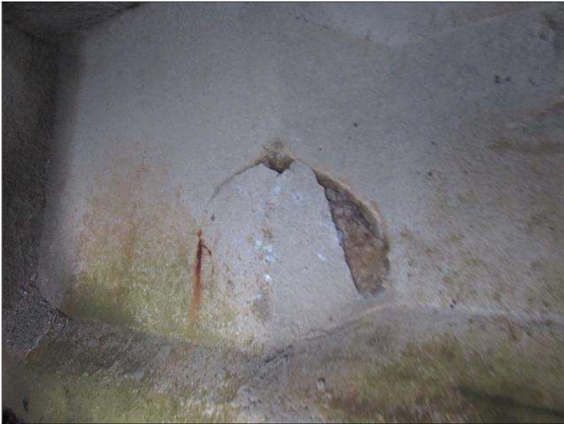
Span 1 Beam 2: 12" DIAMETER DELAMINATION ON RIGHT FACE LOCATED AT END BENT 1
