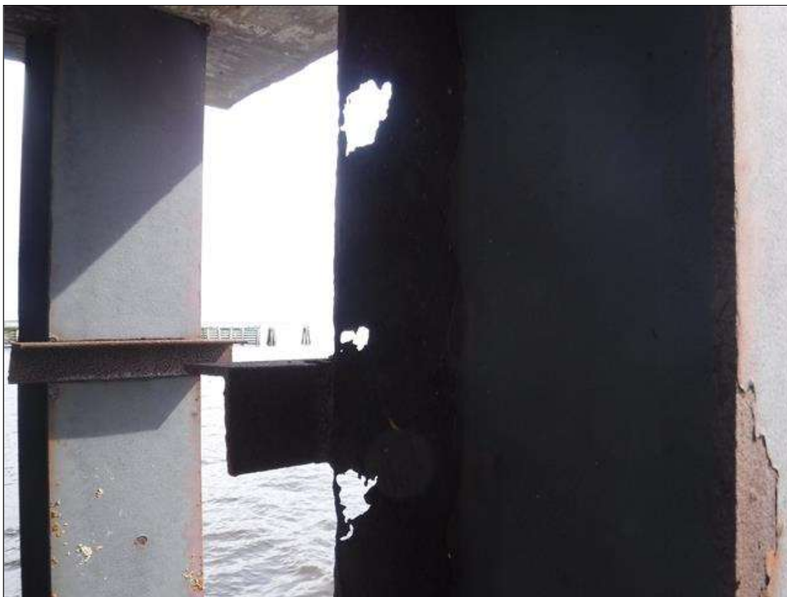
Bent 109 Pile 7: (PAR) 5' RUST SCALE, 0.218" REMAINING, EAST FLANGE, 0.16" REMAINING ON WEST FLANGE, WITH (4) HOLES UP TO 3" X 2" ON EAST FLANGE.
