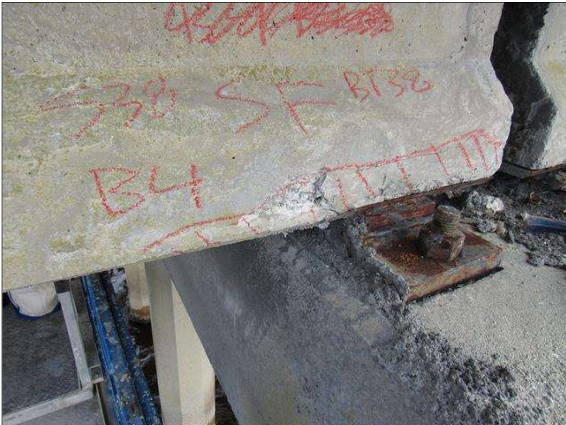
Span 38 Beam 4: 24" X UP TO 4" DELAMINATION ON SOUTH FACE LOCATED AT BENT 38
