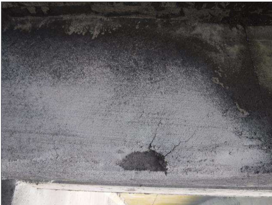
Span 141 Beam 2: 2' X 1' SPALLED PATCHED AREA, WEST FACE, BENT 141 DIAPHRAGM, BETWEEN BEAMS 2 AND 3.
