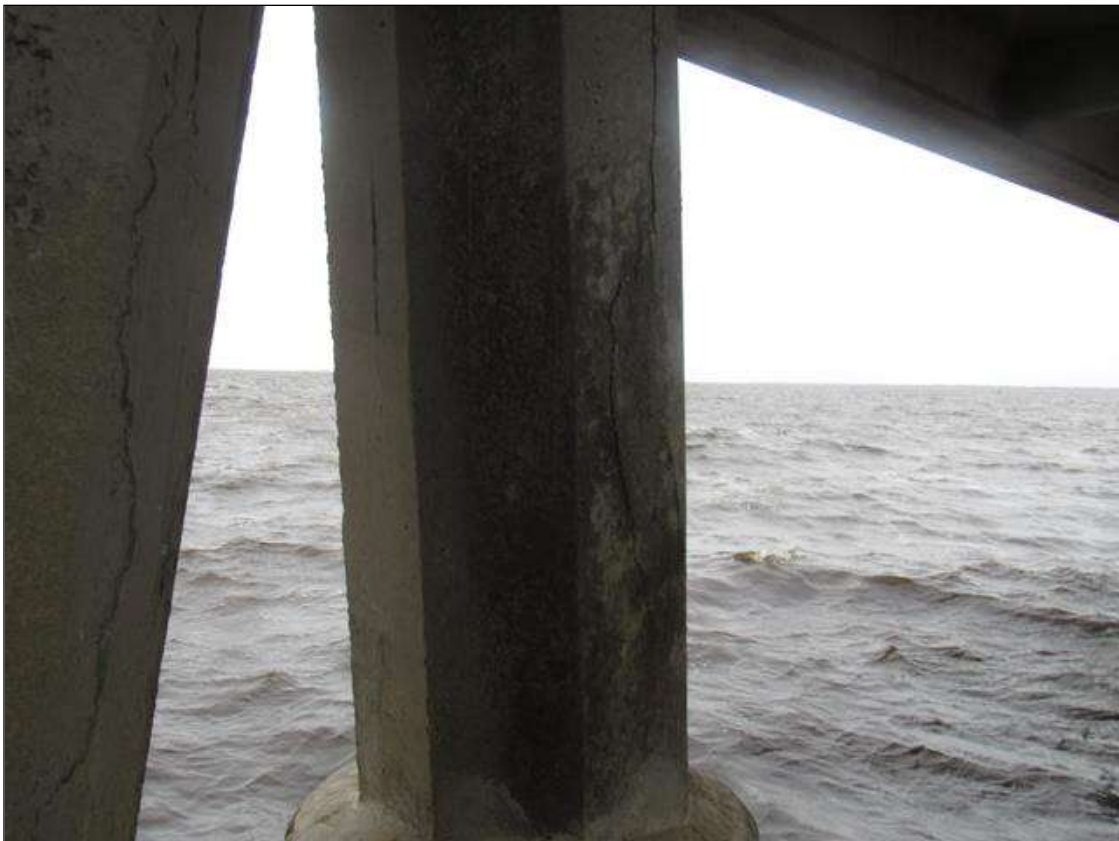
Bent 81 Pile 3: 36" X 8" DELAMINATION, SOUTH FACE, 1' FROM BOTTOM OF CAP.
