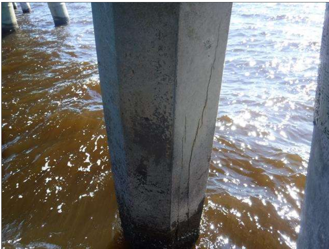
Bent 21 Saved Pile 5: 3' X 1' DELAMINATION, WEST FACE, 8' FROM BOTTOM OF CAP.
