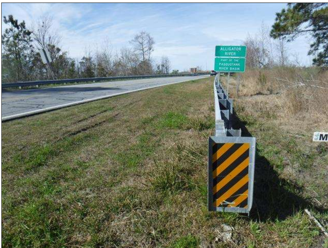
FAR RIGHT GUARDRAIL END UNIT
