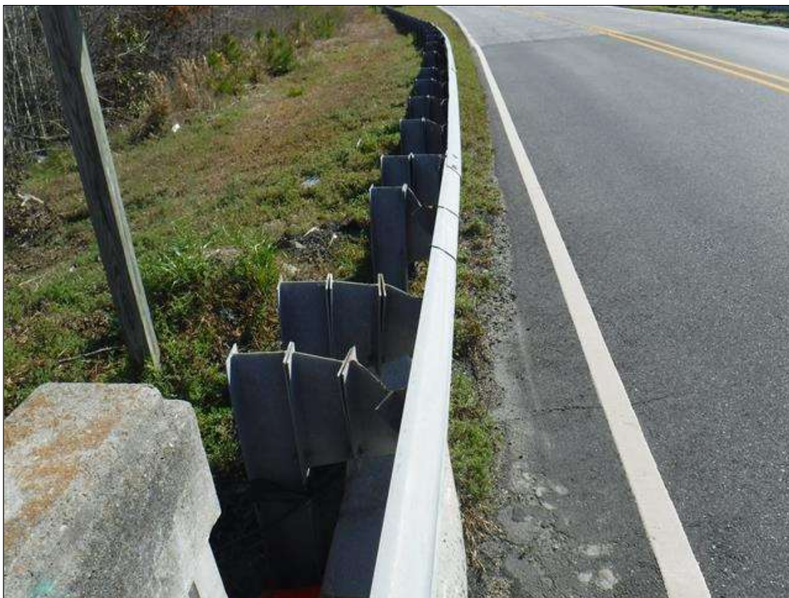
25' OF DAMAGE TO FAR LEFT GUARDRAIL BEGINNING AT END BENT 2
