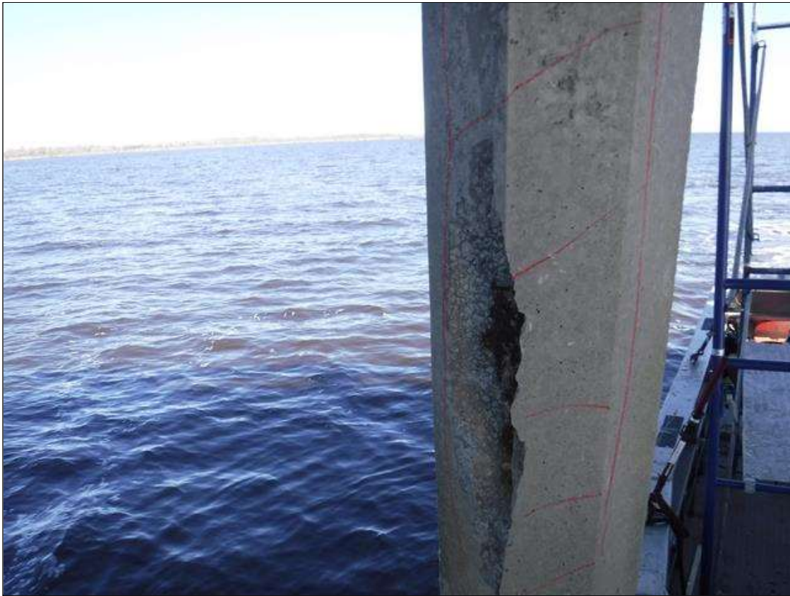
Bent 18 Saved Pile 1: (PAR) 9' X 2' WIDE DELAMINATION WITH 3' X 1' X 3" DEEP SPALL WITH EXPOSED PRESTRESSING ON SOUTH FACE, BEGINNING AT BOTTOM OF CAP AND EXTENDING BELOW WATERLINE. PRESTRESSING HAS 10% SECTION LOSS
