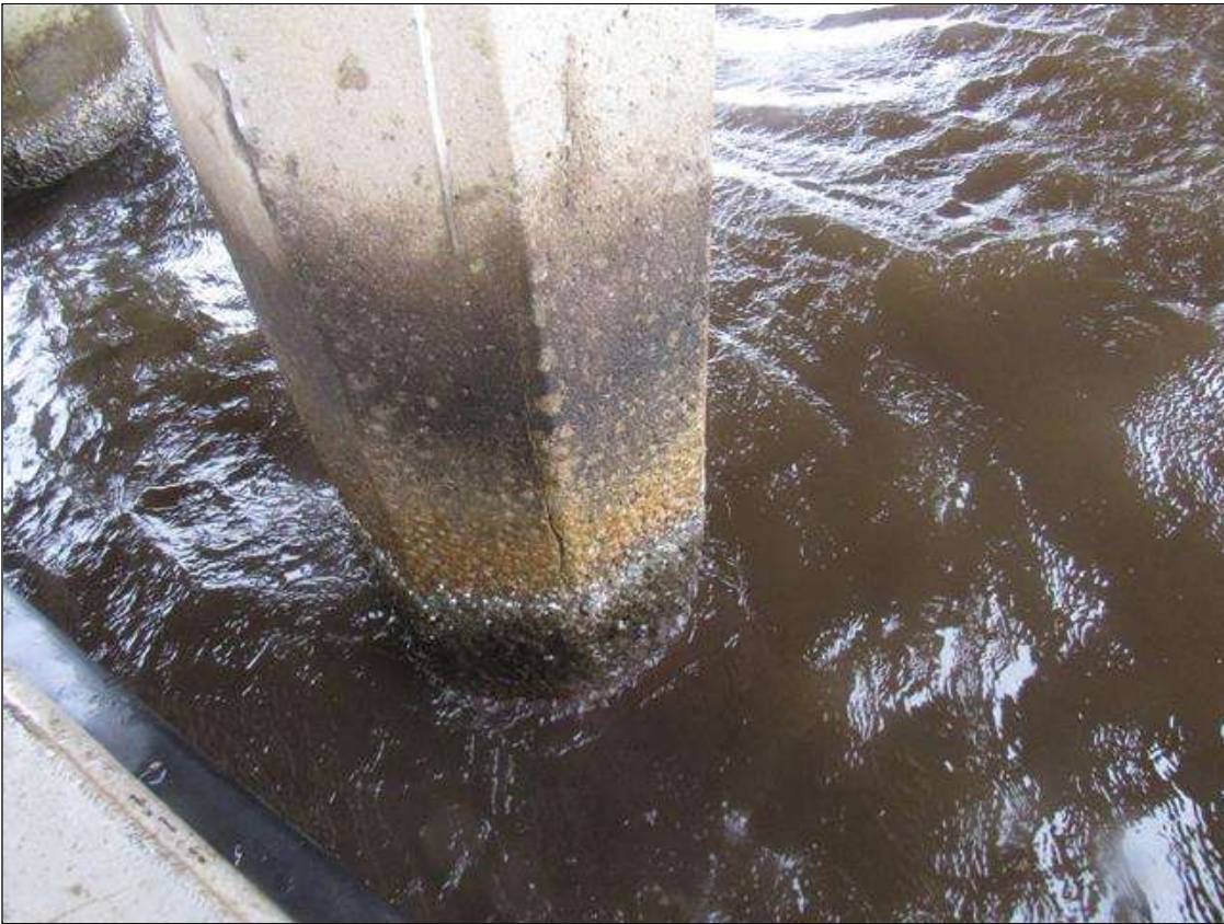
Bent 106 Pile 2: (PAR) (5) UP TO 3' X 1/8" VERTICAL CRACKS, NORTH AND SOUTH FACES, BEGINNING 9' FROM BOTTOM OF CAP, WITH ADJACENT 3' X UP TO 1' DELAMINATION.
