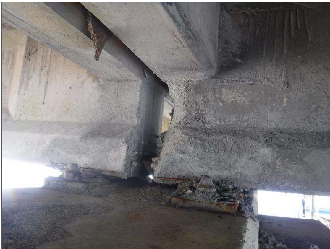
Span 73 Beam 3: (2) UP TO 18" X 12" PATCHED AREAS, NORTH AND SOUTH FACES, AT BENT 73.
