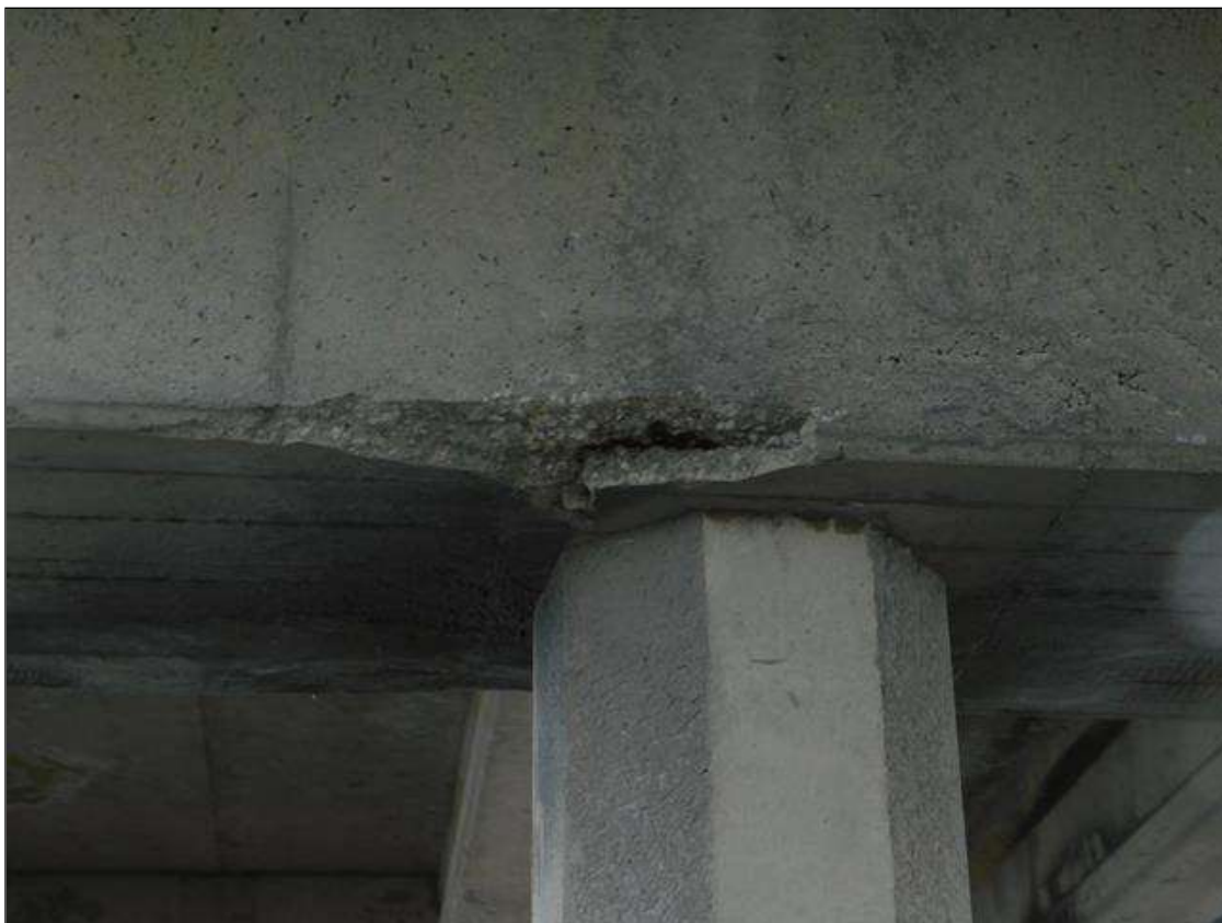
Bent 94 Cap 1: (PAR) 3' X UP TO 11" X 3" SPALL, WITH EXPOSED PRIMARY REINFORCING, BOTTOM OF CAP, BENEATH BEAM 2.
