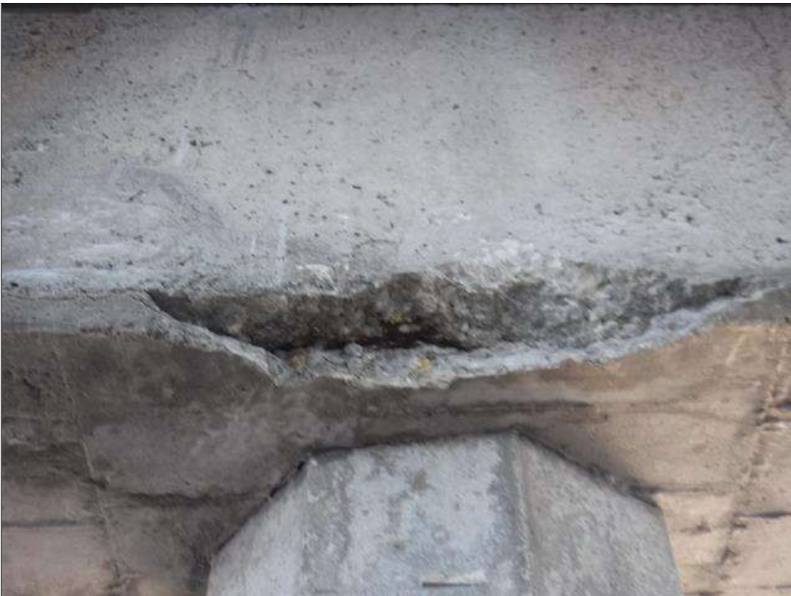
Bent 160 Cap 1: 3' X UP TO 5" X 5" SPALL, WITH EXPOSED PRIMARY REINFORCING, BOTTOM OF WEST FACE, ABOVE PILE 2.
