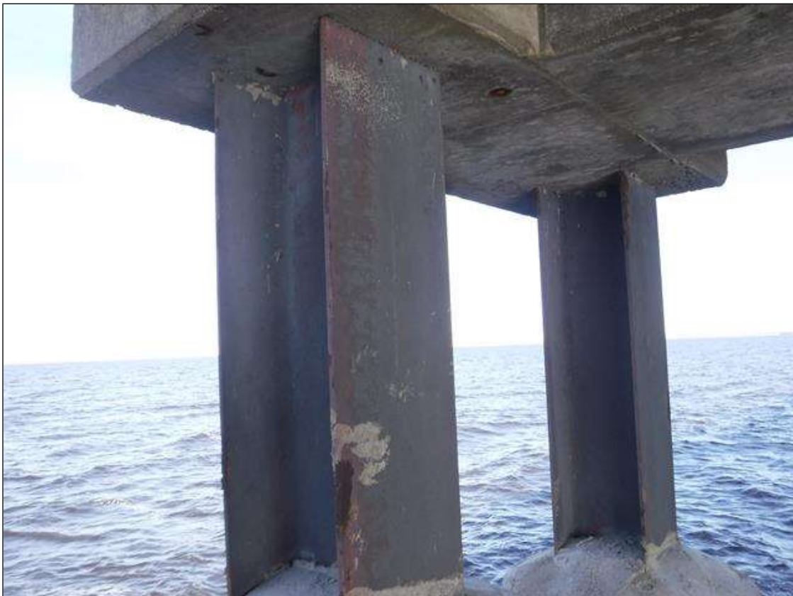
Bent 123 Pile 1: 2' SURFACE RUST, AT RANDOM THROUGHOUT.
