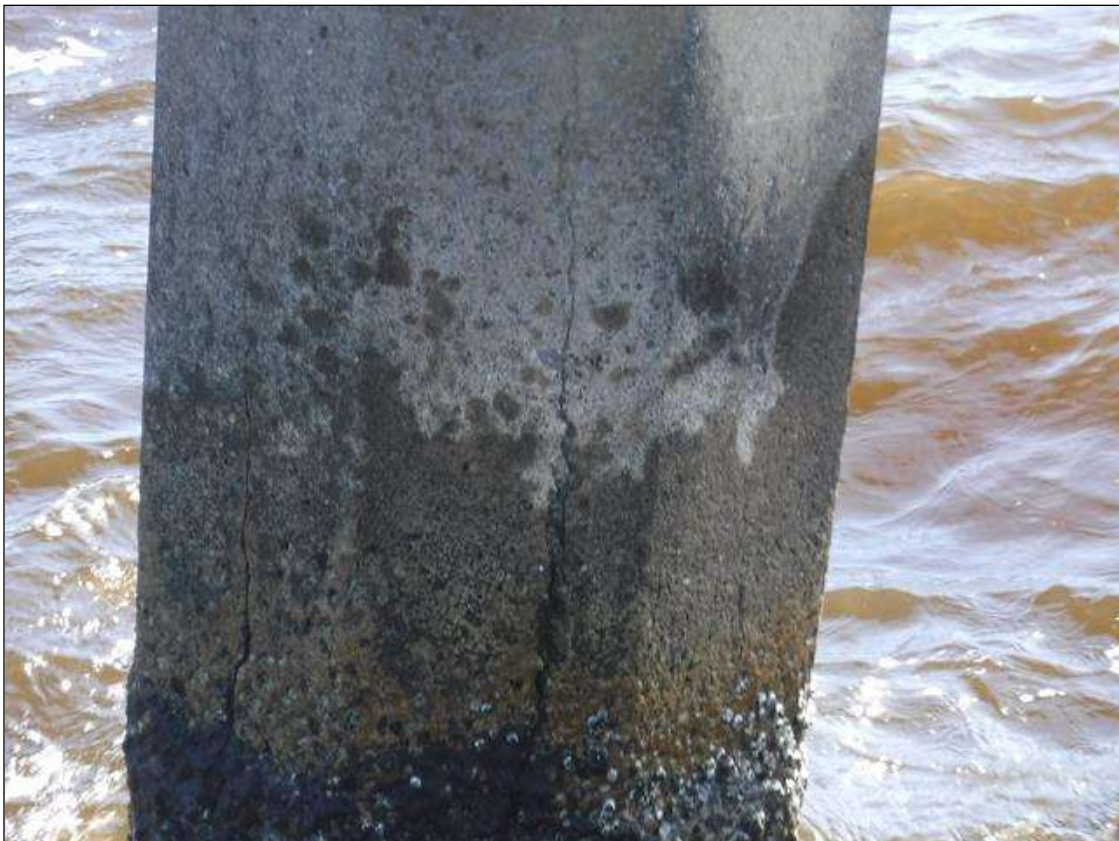
Bent 29 Saved Pile 5: (PAR) HAIRLINE TO 1/8" CRACKS, 8' BELOW CAP, DOWN 5', MULTIPLE FACES. SCALING TO 1" DEEP FROM WATERLINE TO MUDLINE.
