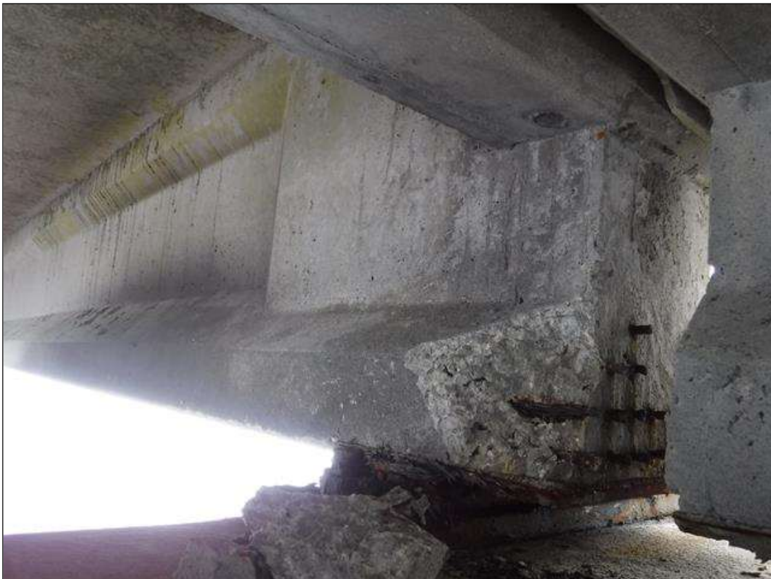
Span 87 Beam 4: (PAR) 10" X 9" X 2" DEEP SPALL WITH EXPOSED STRAND ON NORTH FACE AT BENT 86
