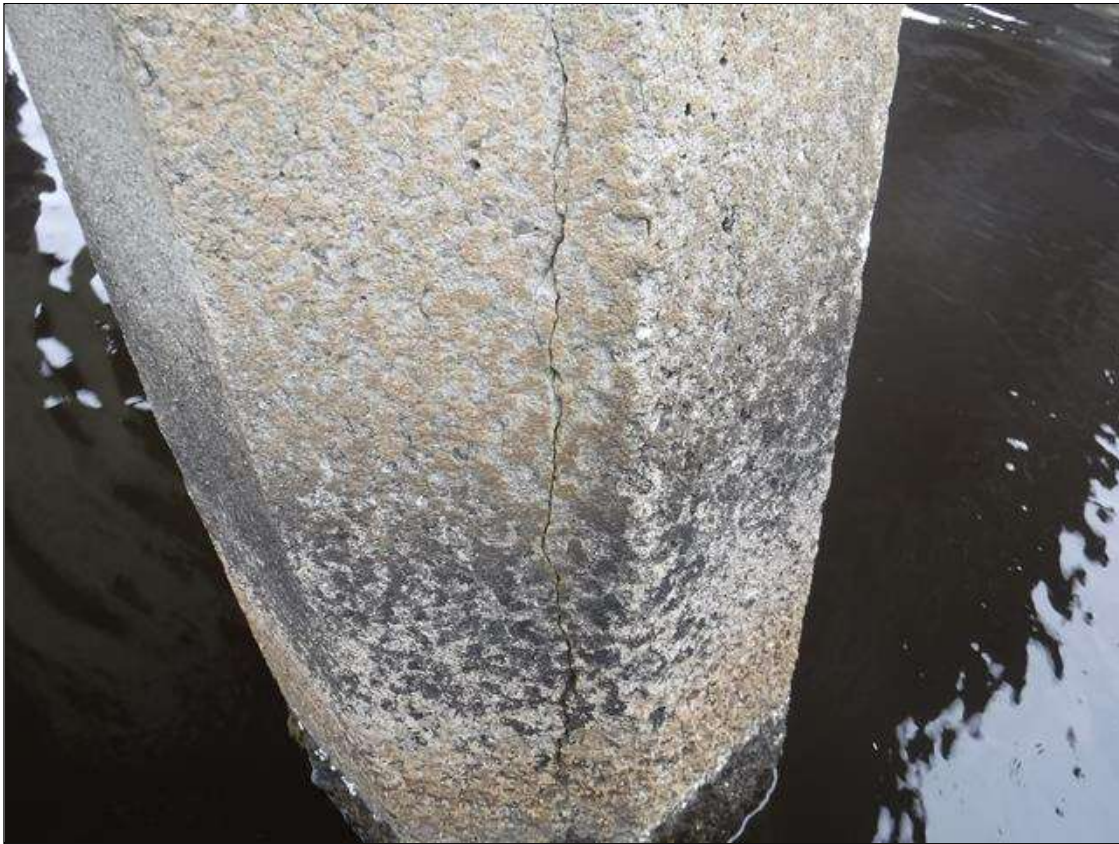
Bent 250 Pile 1: (PAR) UP TO 4' X 0.016" VERTICAL CRACK, NORTH FACE, 7' FROM BOTTOM OF CAP.
