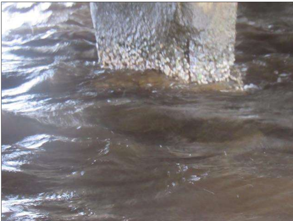
Bent 290 Pile 2: (PAR) 8" X 3" X 3" SPALL, WITH EXPOSED PRIMARY REBAR, NORTHEAST CORNER, 2' FROM BOTTOM OF CAP. REBAR HAS 10% SECTION LOSS
