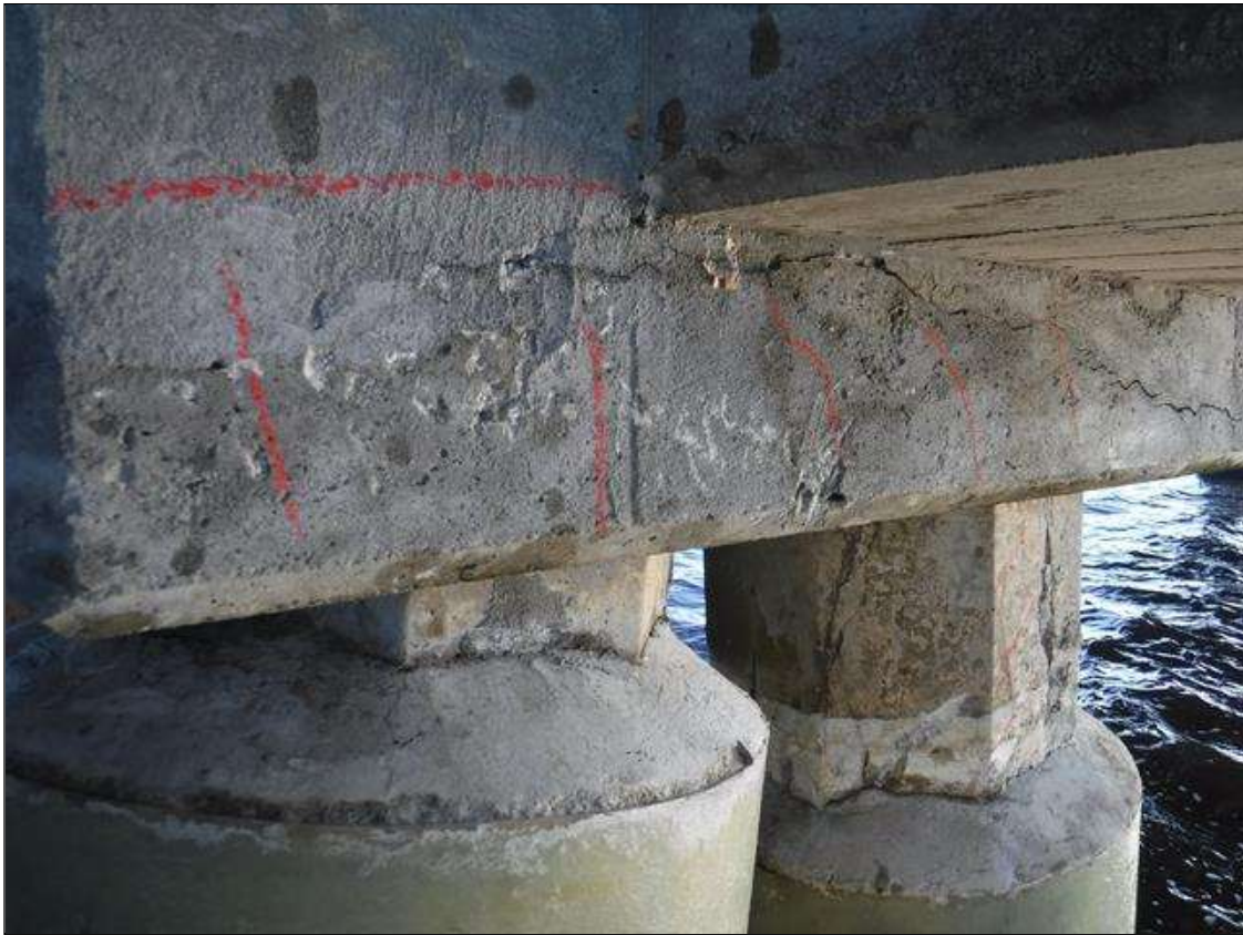
Bent 9 Cap 1: 5' X 8" DELAMINATION, SOUTH FACE OF PILE 4 AND 5 BLOCK-OUT.
