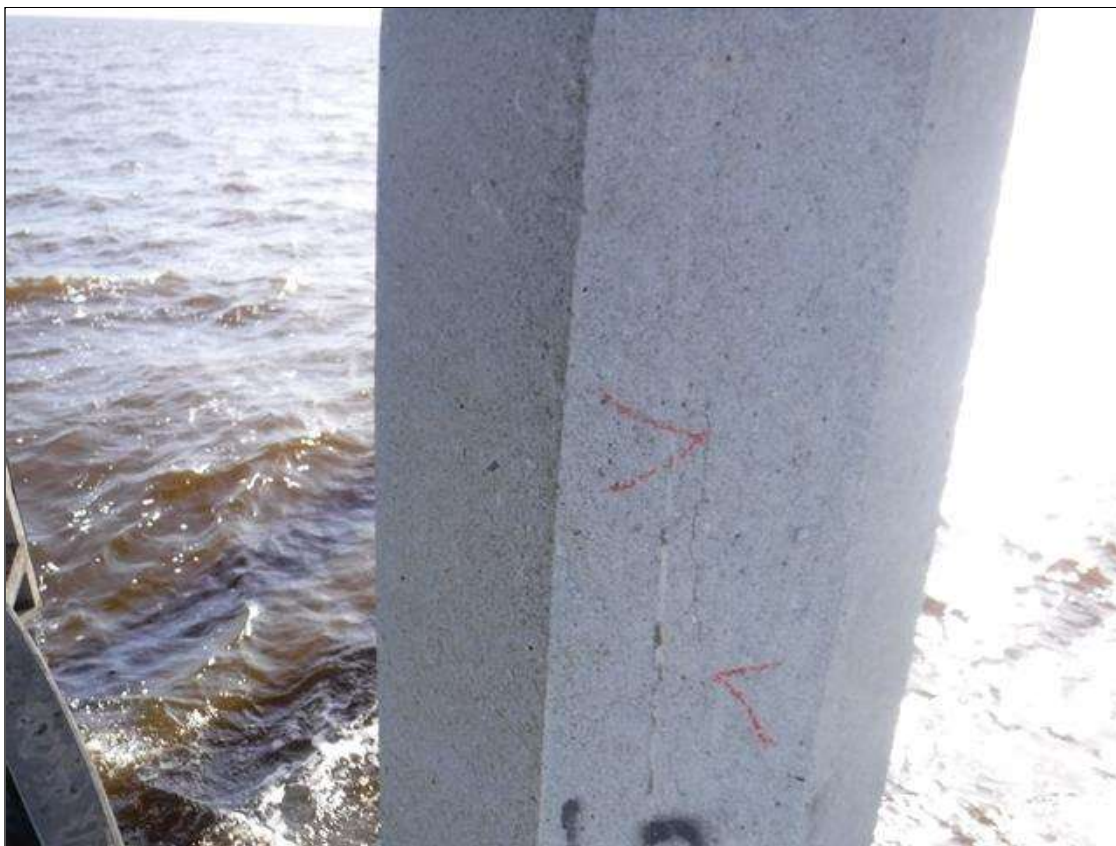
Bent 124 Pile 1: (PAR) 6' X 0.03" VERTICAL CRACK ON NORTH FACE
