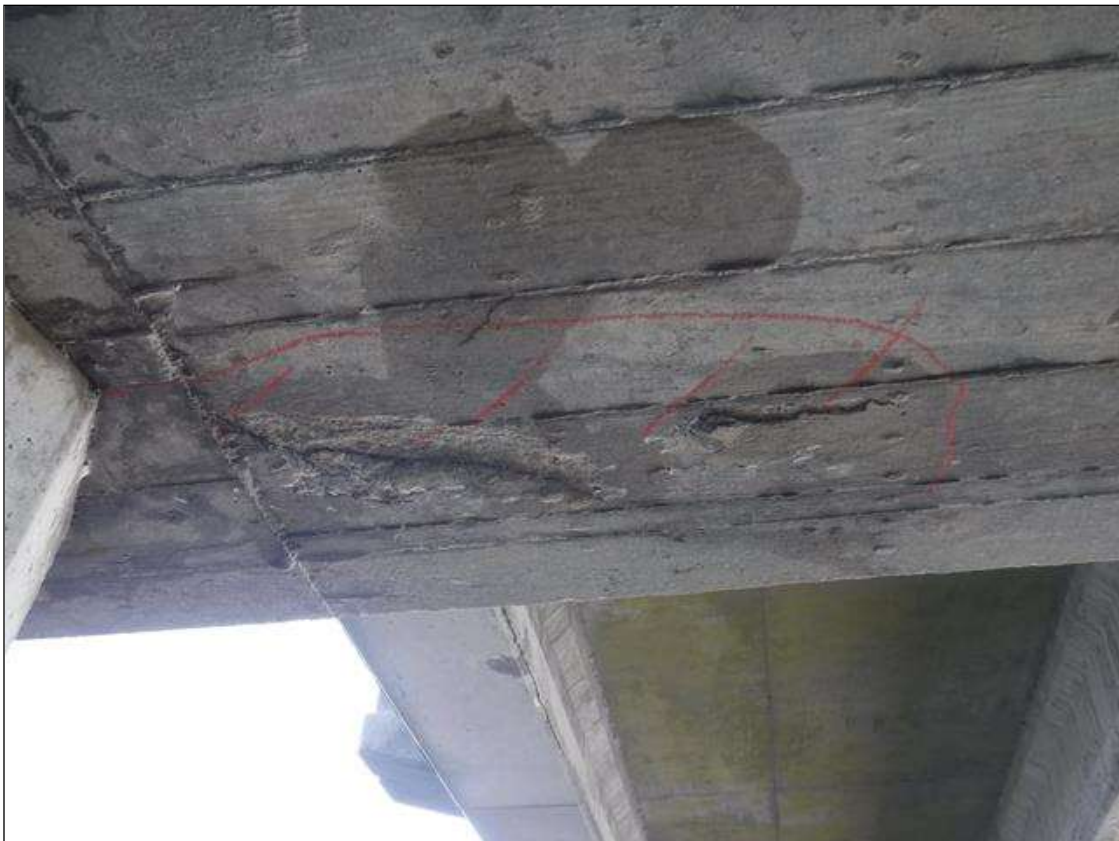
Bent 154 Cap 1: 3' X 12" AREA OF DELAMINATION ON BOTTOM OF CAP, AT PILE 1.
