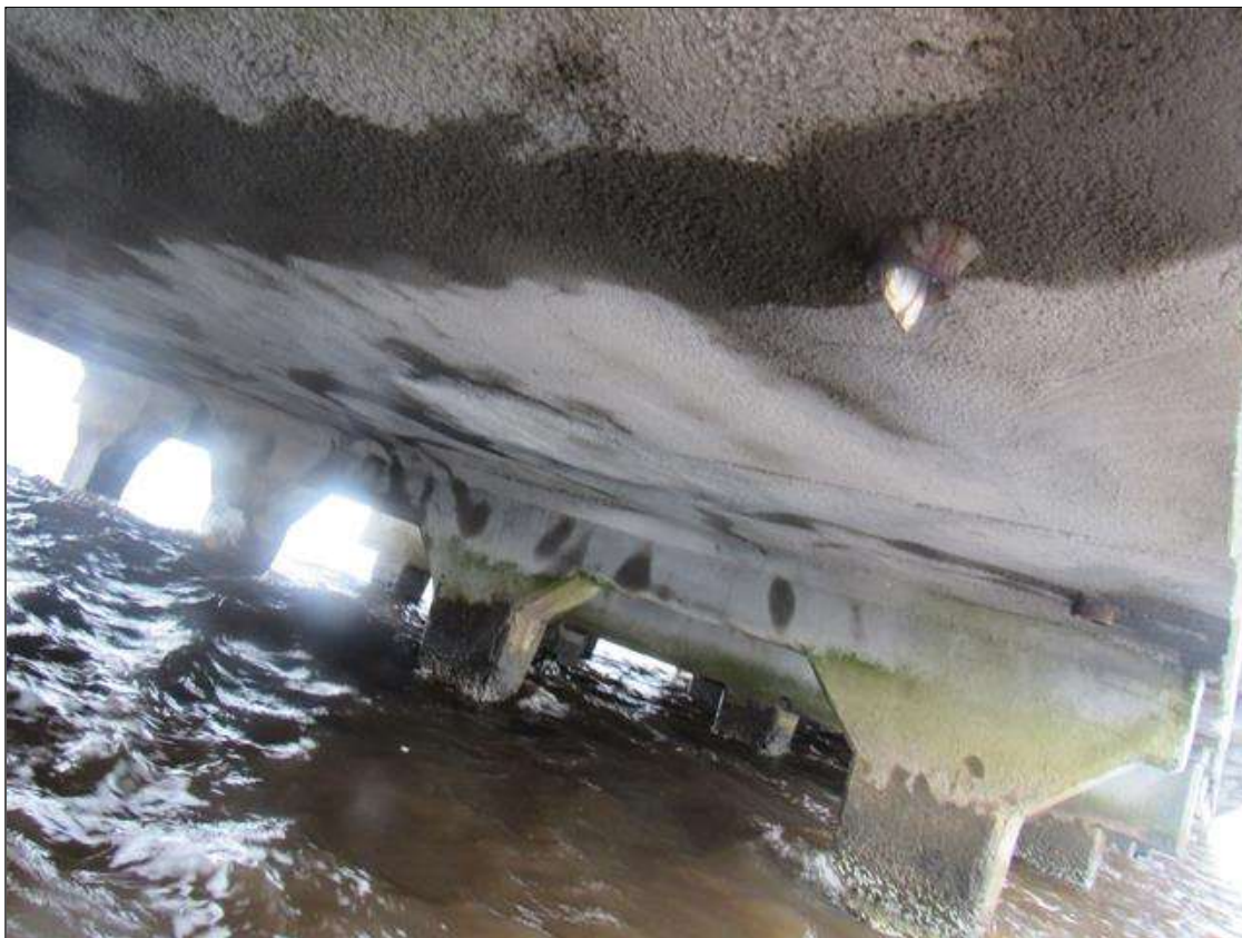
Span 291 Deck: 180 SF OF PATCHED AREA, AT RANDOM THROUGHOUT DECK UNDERSIDE.
