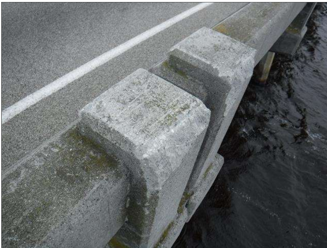
Span 239 Left Bridge Rail: (8) UP TO 10" X 6" X 3" SPALLS AT TOP LEFT CORNER LOCATED ON POSTS 1 AND 3 THROUGH 9
