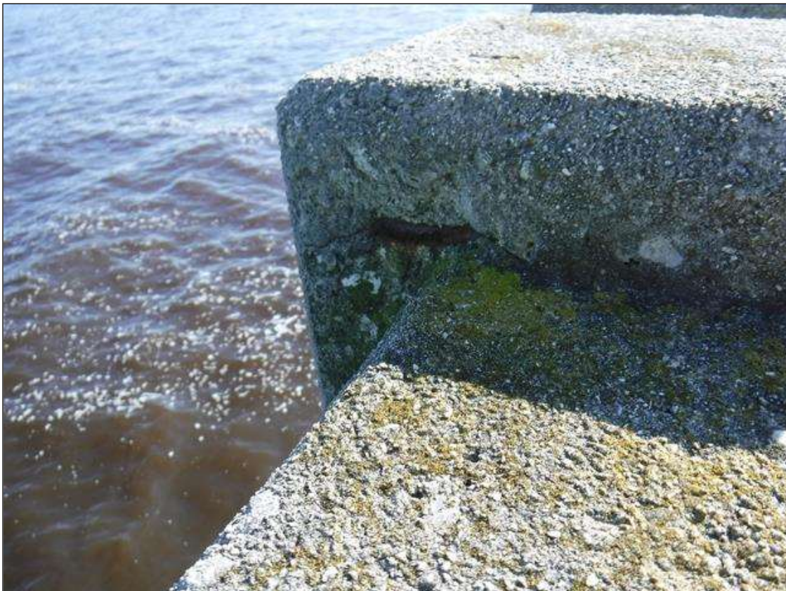
Span 8 Left Bridge Rail: 3" X 2" X 3/4" SPALL WITH EXPOSED REBAR ON NEAR FACE LOCATED AT LAST END POST
