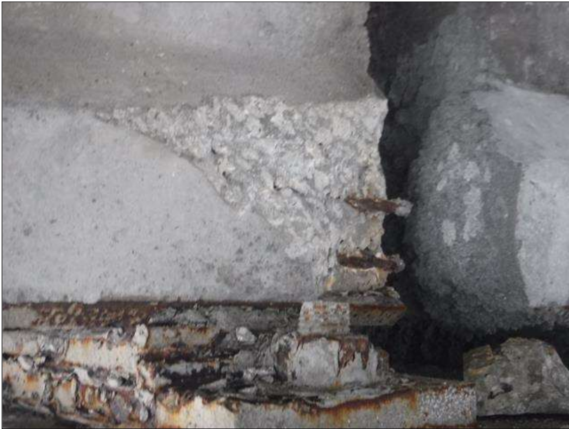
Span 175 Beam 2: (PAR) 12" X 10" X 1" DEEP SPALL WITH EXPOSED STRANDS ON NORTH FACE AT BENT 174
