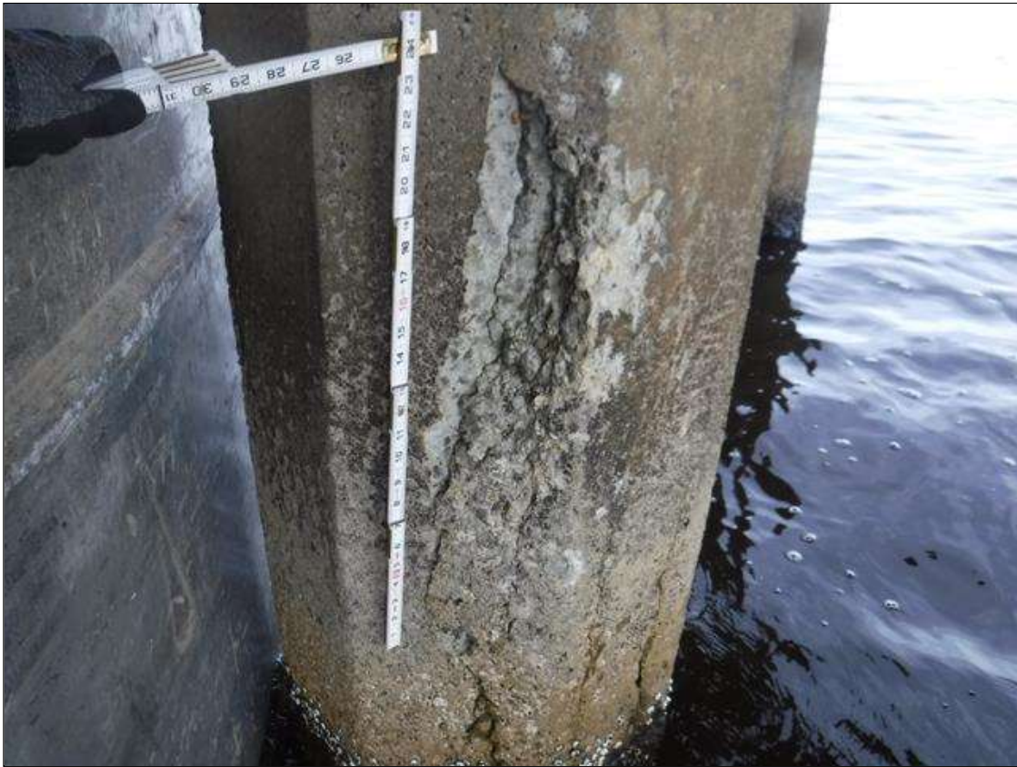
Bent 227 Pile 2: (PAR) 3' X 10" X 1" DEEP SPALL, SOUTH FACE, 8' FROM BOTTOM OF CAP.
