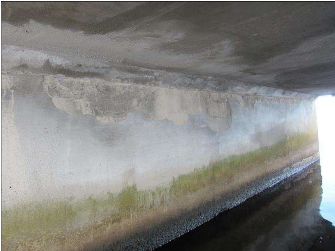
Bent 277 Cap 1: (PAR) 12' LONG X 18" HIGH X 2.5" DEEP SPALL LOCATED ON TOP EDGE OF EAST FACE, BEGINNING 8' FROM SOUTH END. SPALL CAUSING LOSS OF BEARING AREA IN SLAB.
