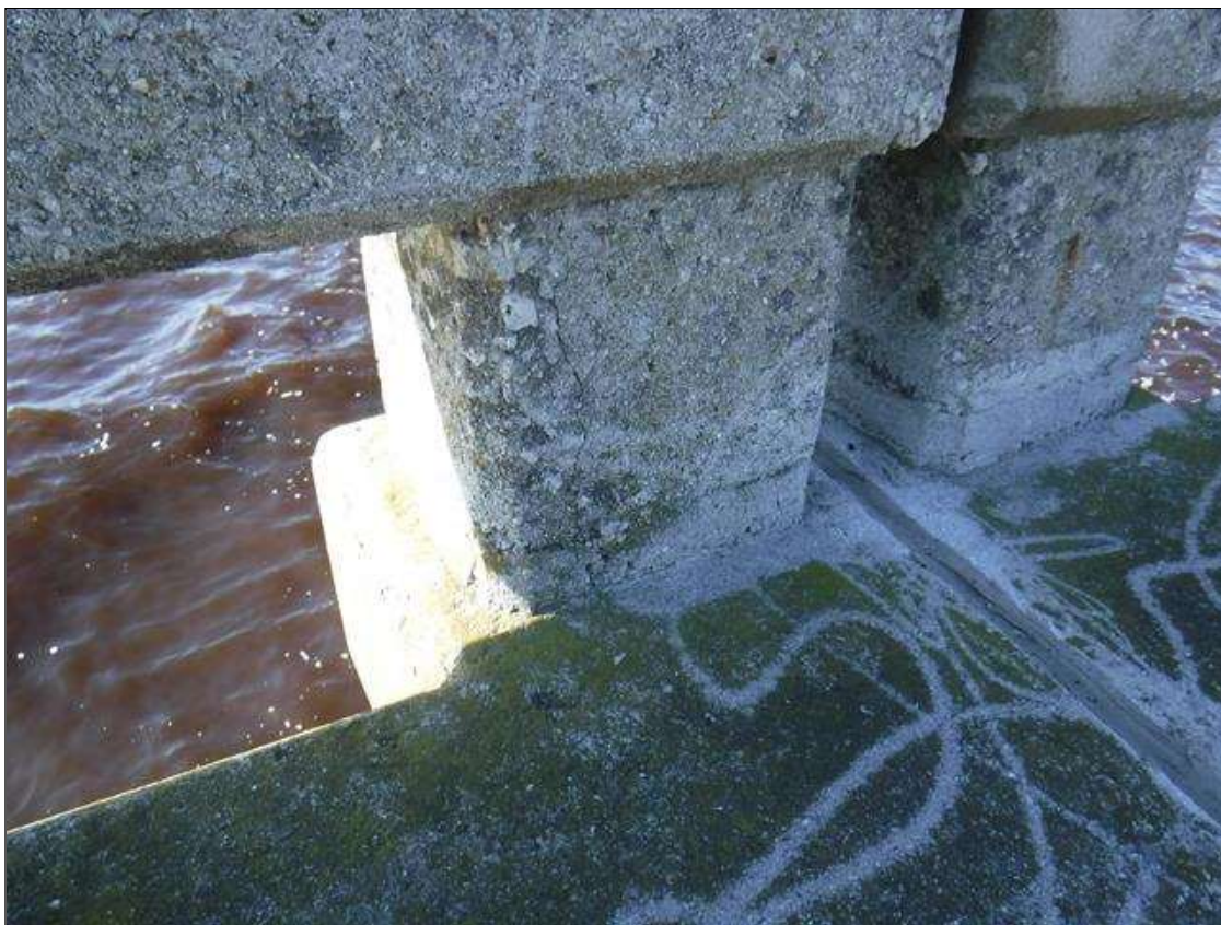
Span 3 Right Bridge Rail: 8" X UP TO 1/32" VERTICAL CRACK, NORTH FACE, RAIL POST AT BENT 2.
