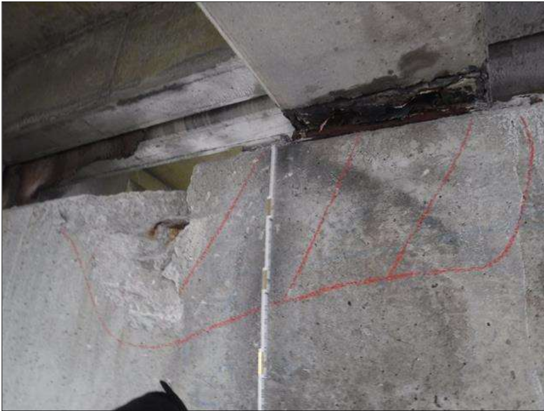
Bent 192 Cap 1: (PAR) 4' X 2' DELAMINATION WITH 18" DIAMETER X 6" DEEP SPALL WITH EXPOSED REBAR IN EAST FACE BELOW BEAM 3
