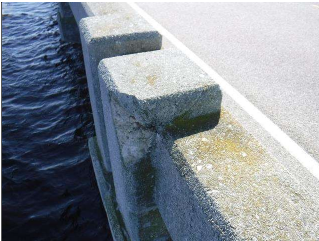
Span 154 Left Bridge Rail: 8" X 5" X 7" SPALL WITH EXPOSED REBAR AT TOP LEFT CORNER LOCATED ON POST 6
