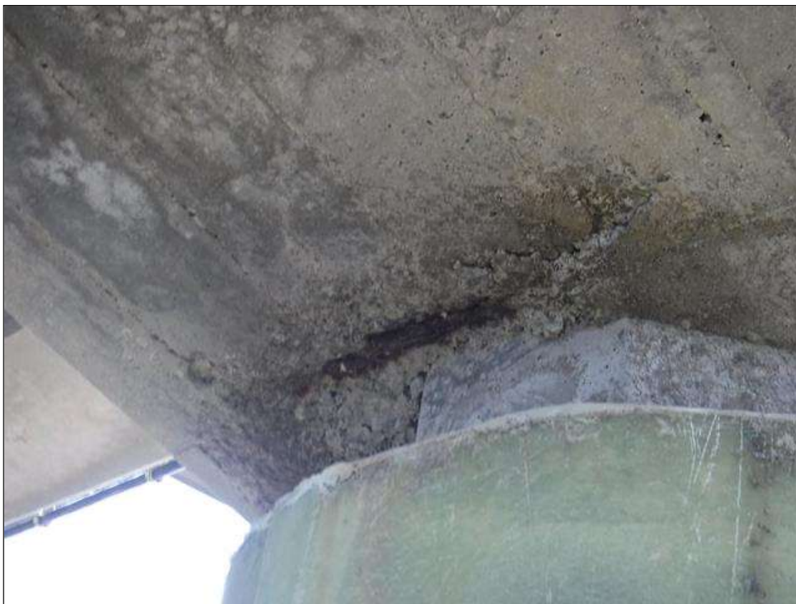
Bent 22 Cap 1: (PAR) 12" X 24" X 4" SPALL, WITH EXPOSED REINFORCING, BOTTOM FACE, BENEATH BEAM 4. REBAR HAS 10% SECTION LOSS
