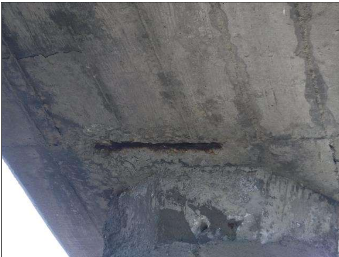
Bent 118 Cap 1: 2' X 6" X 1" DEEP SPALL WITH EXPOSED REBAR ON BOTTOM FACE AT PILE 4
