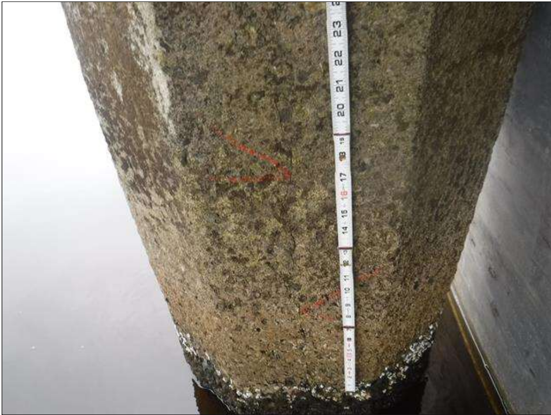
Bent 237 Pile 4: (PAR) (2) UP TO 3' X 0.03" VERTICAL CRACKS, BEGINNING 7' FROM BOTTOM OF CAP, AT RANDOM THROUGHOUT.
