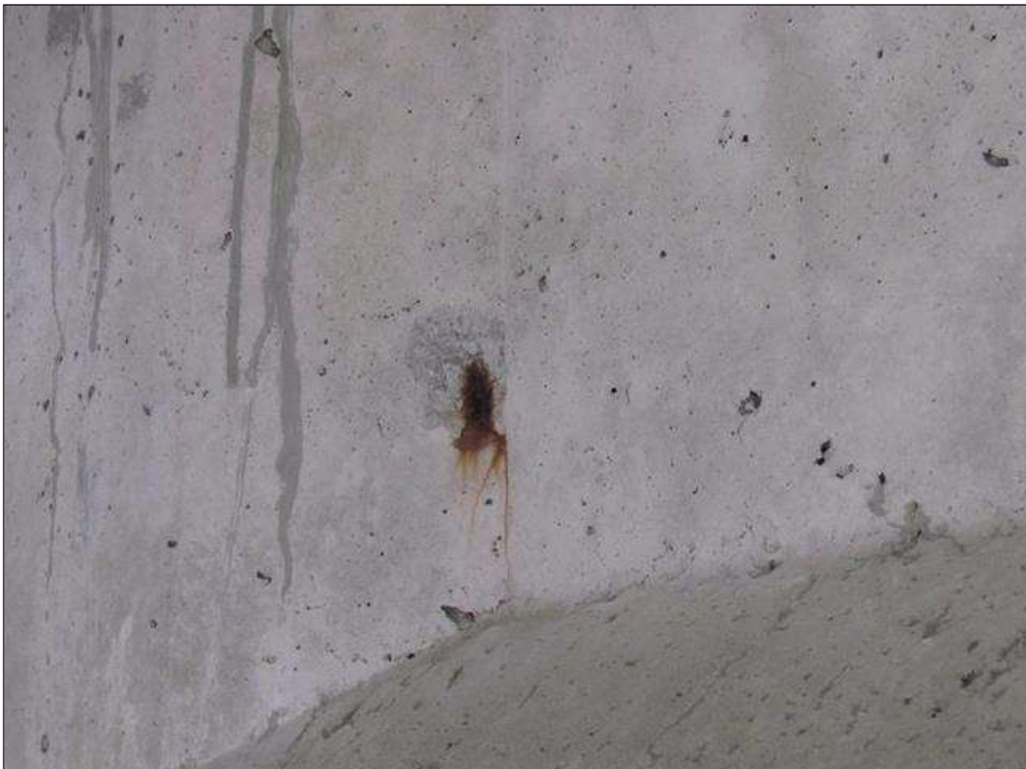
Span 53 Beam 3: 2" DIAMETER X 1/4" DEEP SPALL WITH EXPOSED REBAR, NORTH FACE, 2' FROM BENT 53.
