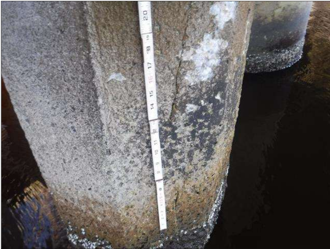
Bent 211 Pile 5: (PAR) UP TO 2' X 0.010" VERTICAL CRACKS, NORTH FACE, 8' FROM BOTTOM OF CAP, WITH ADJACENT 2' X 1' DELAMINATION.
