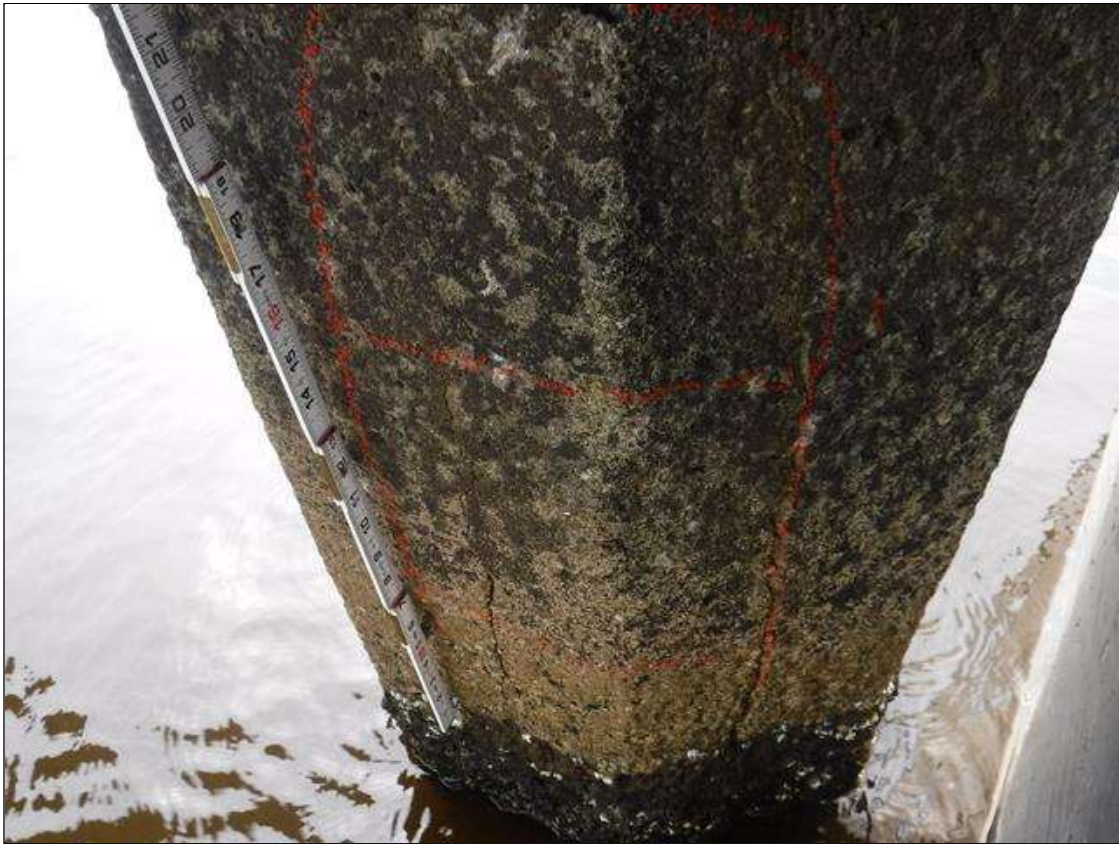
Bent 229 Pile 4: (PAR) (4) UP TO 6' X 0.03" VERTICAL CRACKS, AT RANDOM THROUGHOUT, BEGINNING 5' FROM BOTTOM OF CAP, WITH ADJACENT 2' X 1' DELAMINATION ON NORTH AND EAST FACE
