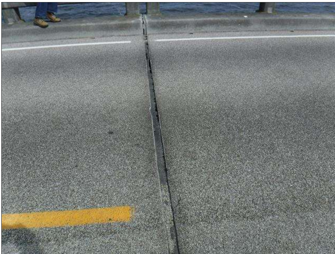
Expansion Joint 186 : 30' ADHESION FAILURE ALONG ENTIRE JOINT LOCATED OVER BENT 186
