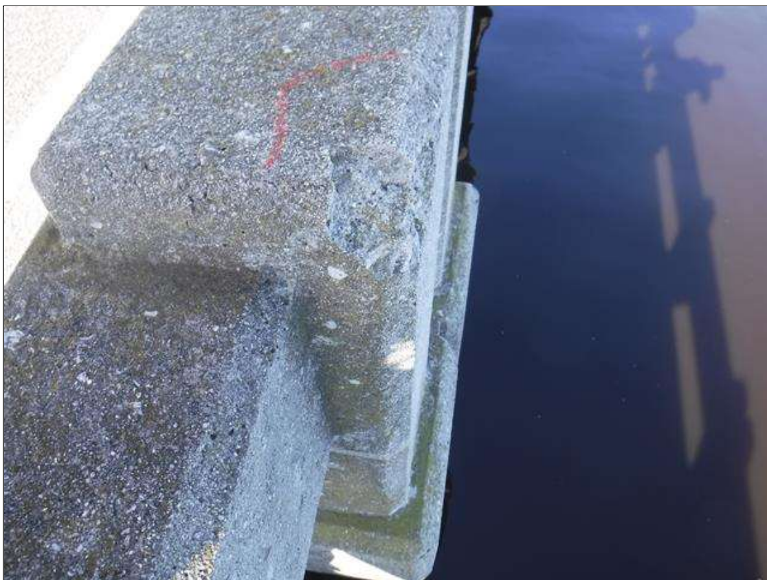
Span 268 Left Bridge Rail: 4" X 3" X 4" SPALL ON LEFT FACE ON POST 7
