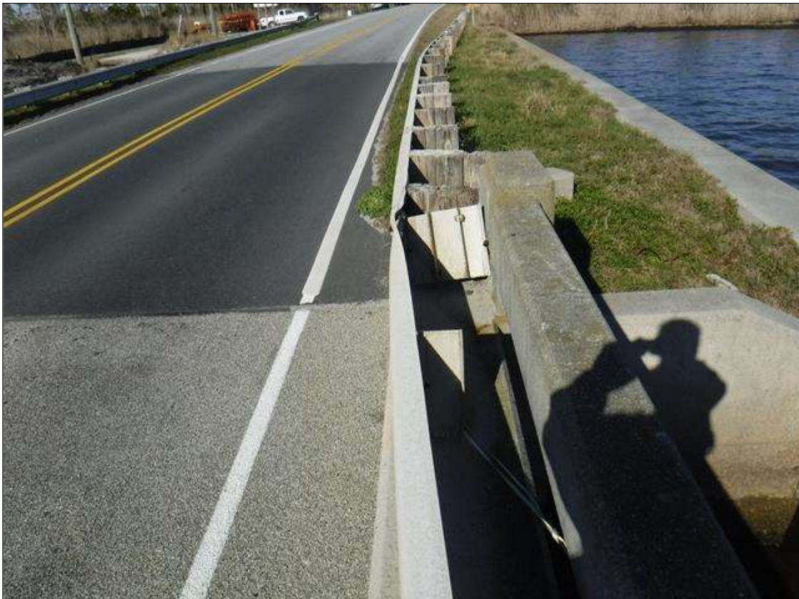
Span 1 Left Bridge Rail: 3' OF DAMAGE TO LEFT RAIL ATTACHMENT
