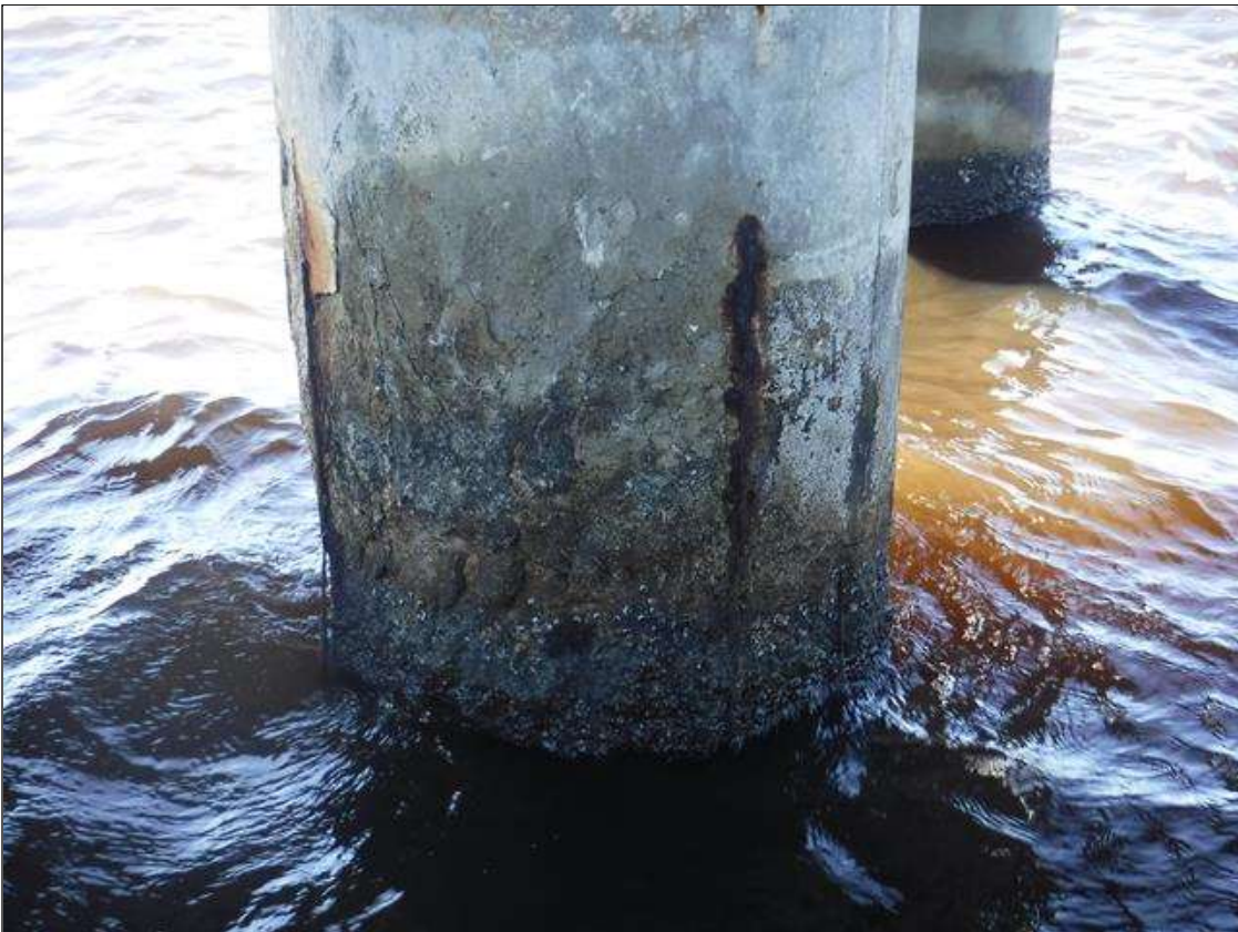
Bent 11 Saved Pile 3: (PAR) 4' X 2' X UP TO 1.5" SPALL ON PILE JACKET, WITH EXPOSED REINFORCING WITH COMPLETE SECTION LOSS, NORTH FACE, 5' FROM BOTTOM OF CAP.
