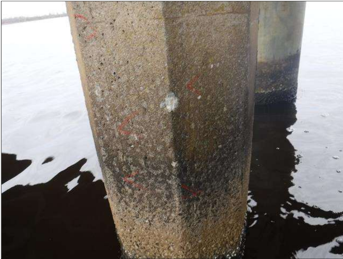
Bent 254 Pile 2: (PAR) (4) UP TO 4' X 0.02" VERTICAL CRACKS, EAST AND NORTH FACES, 7' FROM BOTTOM OF CAP, WITH UP TO 4' X 1' DELAMINATIONS.
