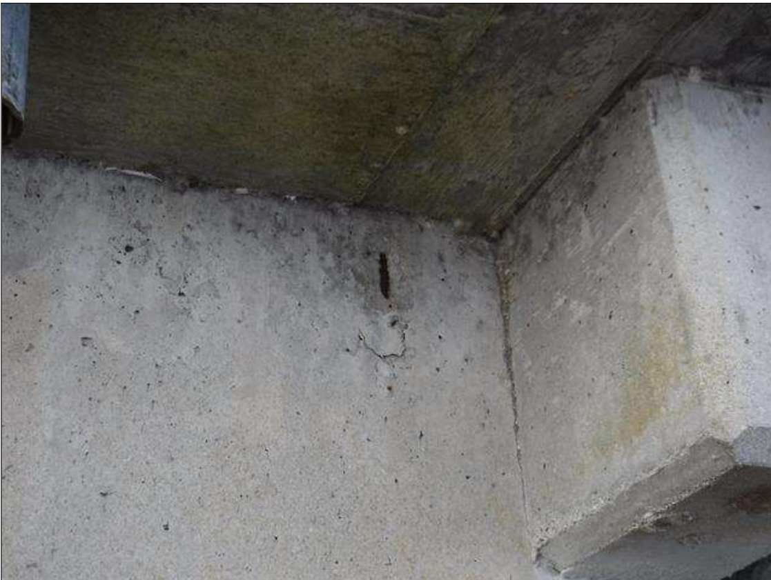
Span 203 Beam 1: 3" X 4" X 1/2" SPALL, WITH EXPOSED REINFORCING, NORTH FACE, AT BENT 202.
