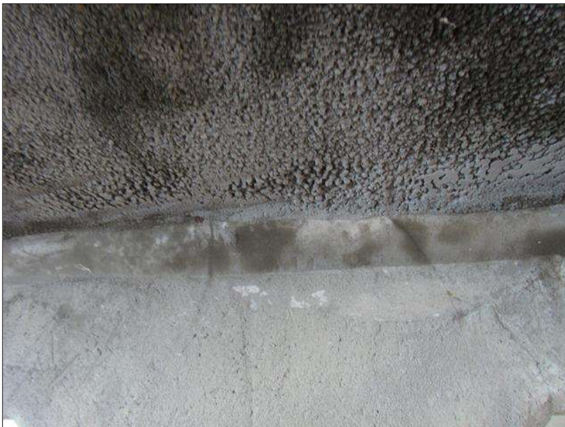
Span 279 Deck: 12" X 6" PATCHED AREA ON DECK UNDERSIDE, NEAR BENT 280.
