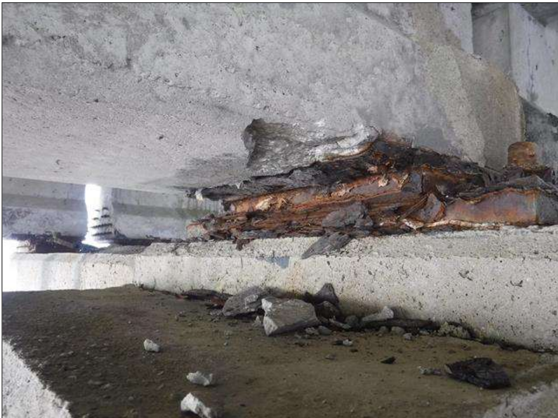
Span 78 Beam 3: 6" X 6" X 1/2" DEEP SPALL, NORTH FACE, AT BENT 77.
