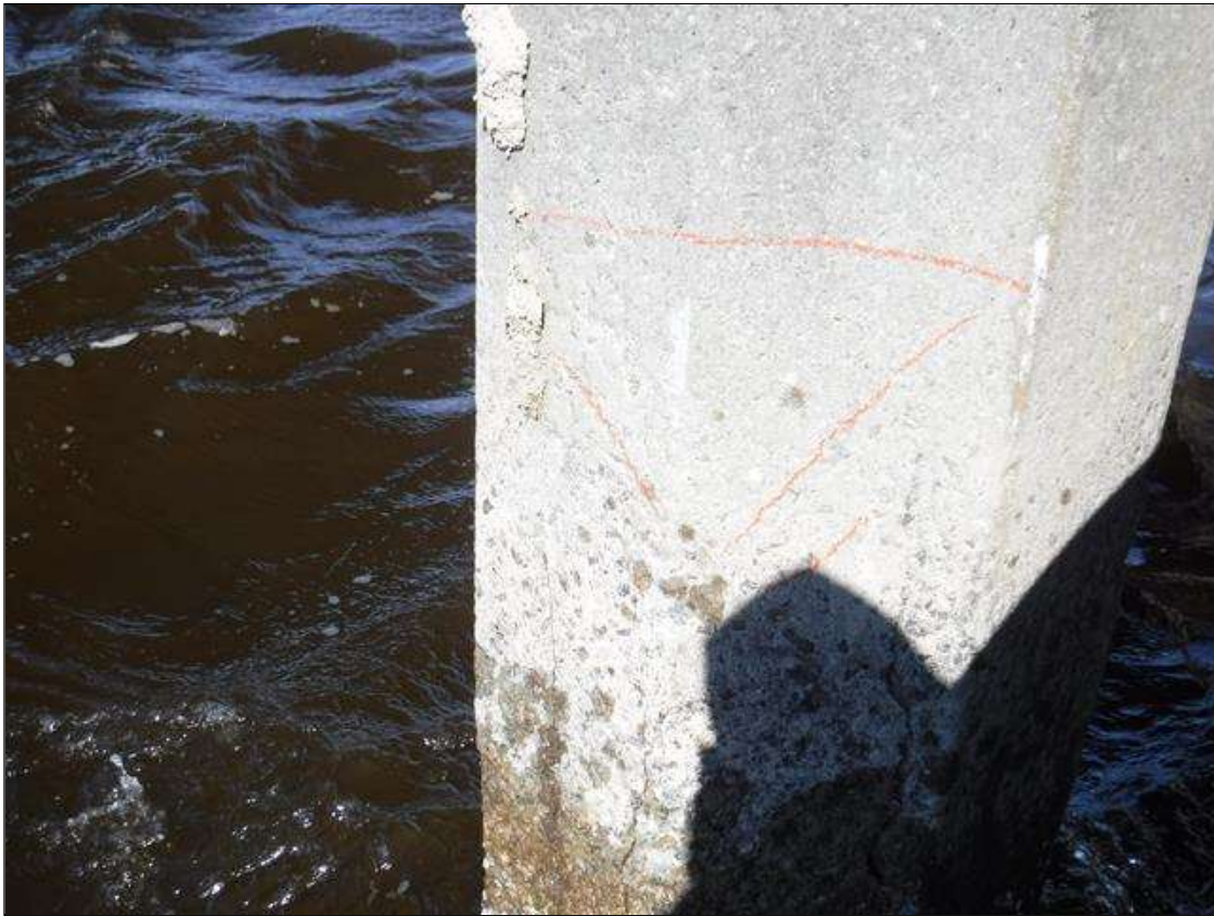
Bent 19 Saved Pile 4: 2' X 1' DELAMINATION, SOUTH FACE, 8' FROM BOTTOM OF CAP.
