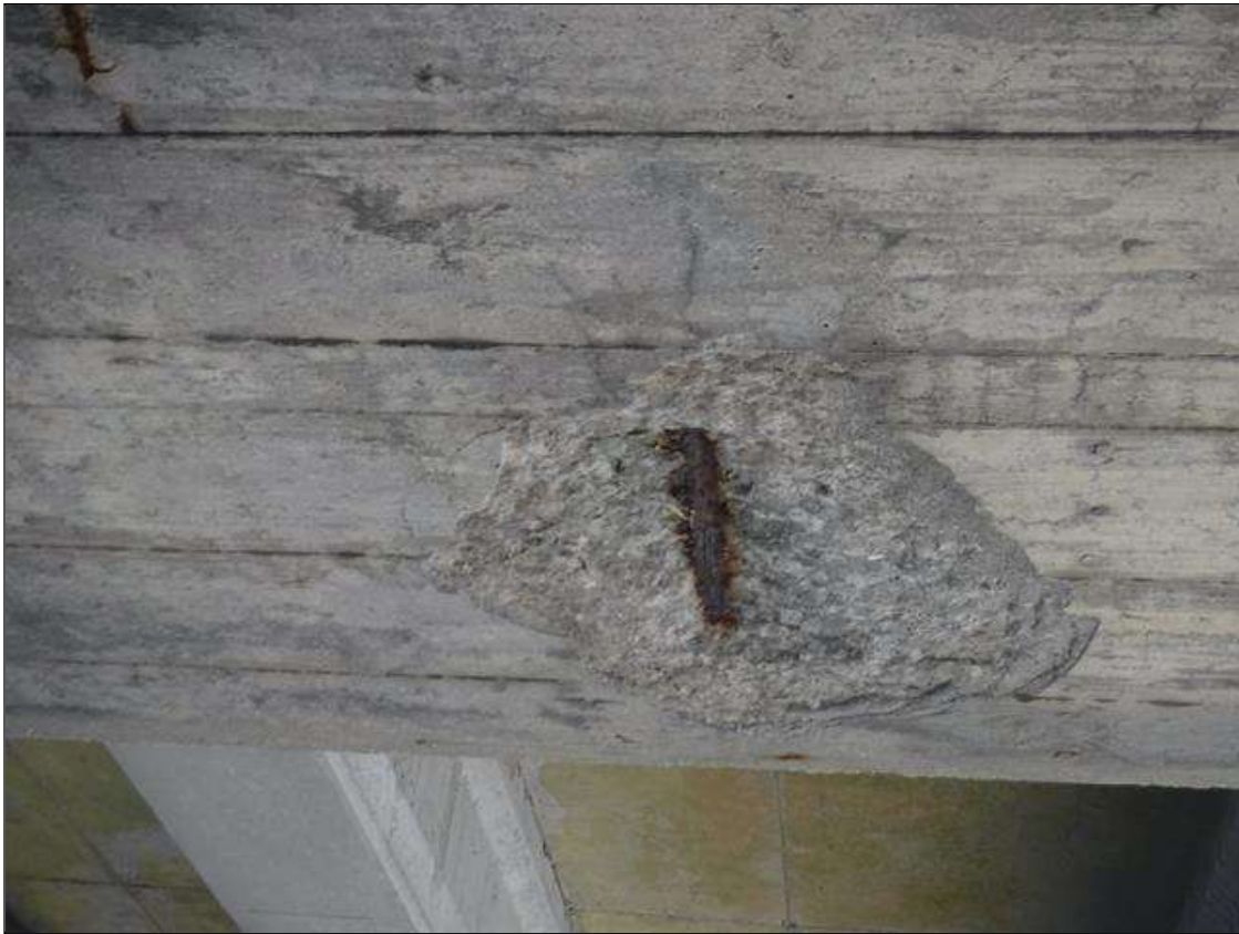
Bent 220 Cap 1: (PAR) 16" DIAMETER X 3/4" DEEP SPALL WITH EXPOSED REINFORCEMENT IN BOTTOM OF CAP BETWEEN PILS 3 AND 4. REBAR HAS 10% SECTION LOSS.
