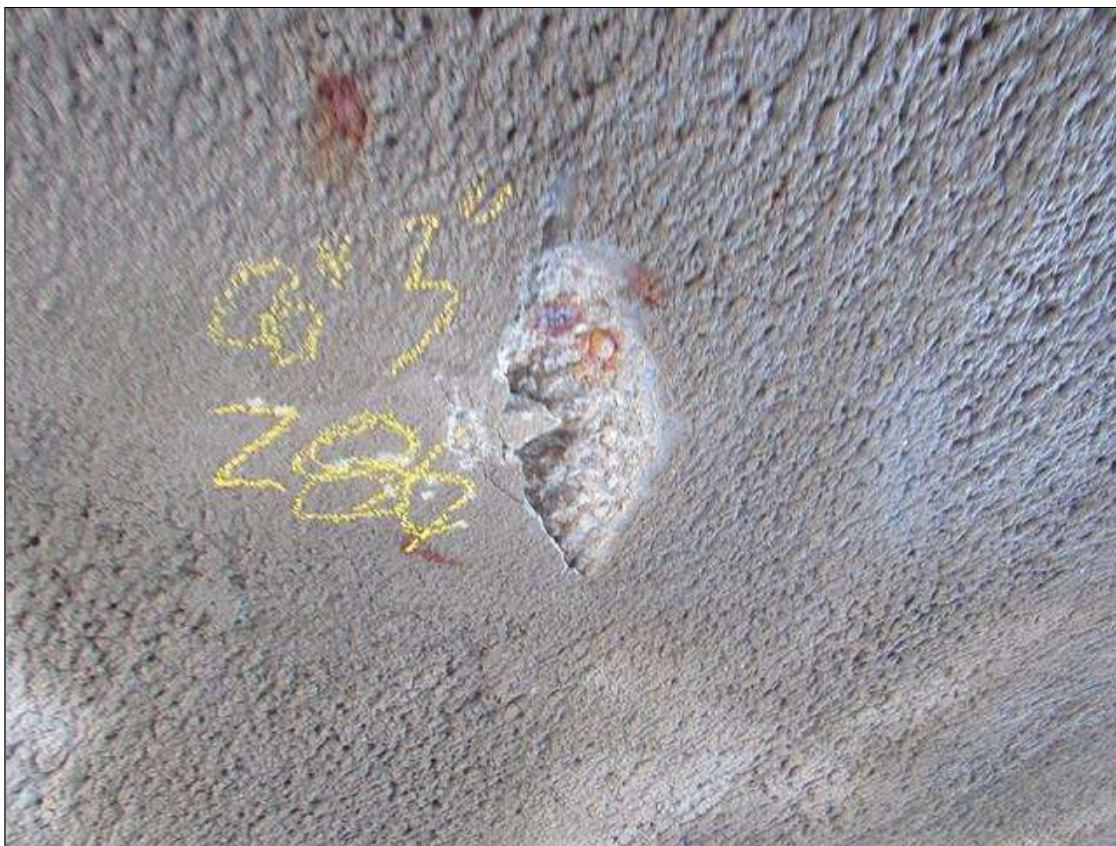
Span 286 Deck: 8" X 3" X 1/2" DEEP SPALL ON BOTTOM FACE LOCATED AT MID-SPAN NEAR PILE 2
