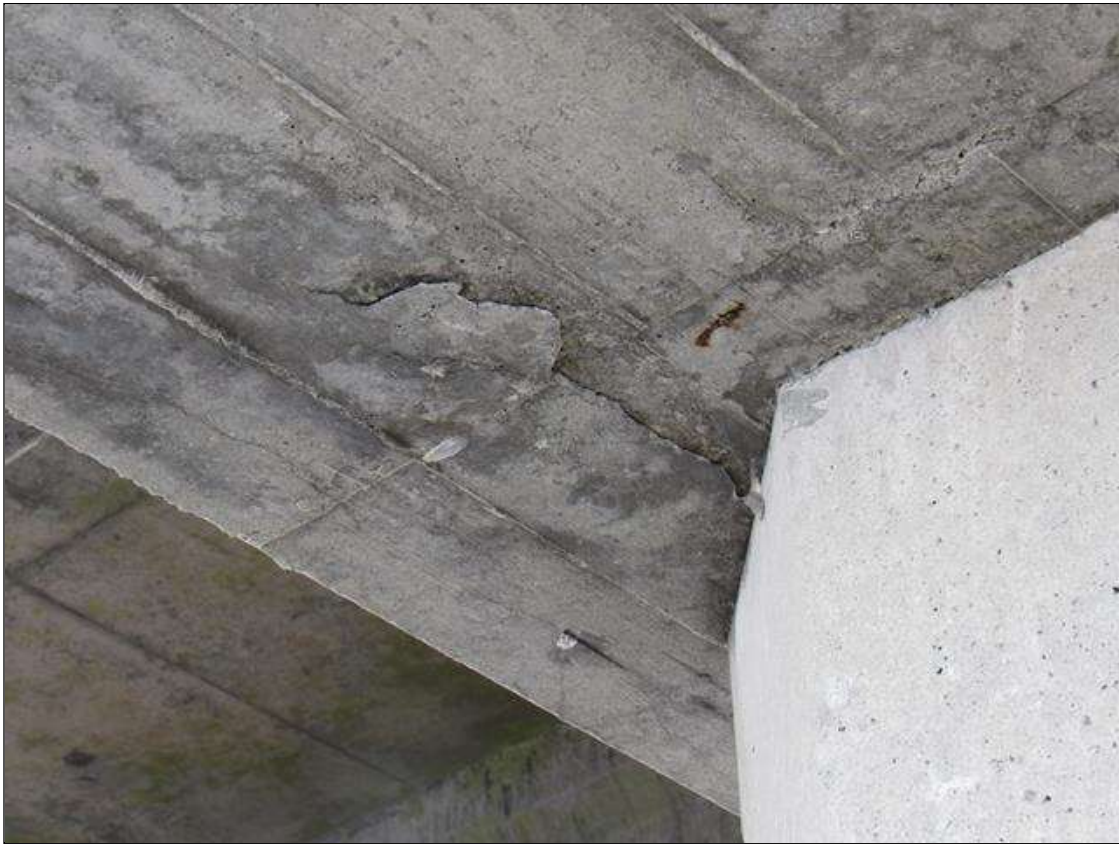
Bent 31 Cap 1: 8" X 14" DELAMINATION ON EAST FACE AT BOTTOM OF CAP NEAR PILE 3
