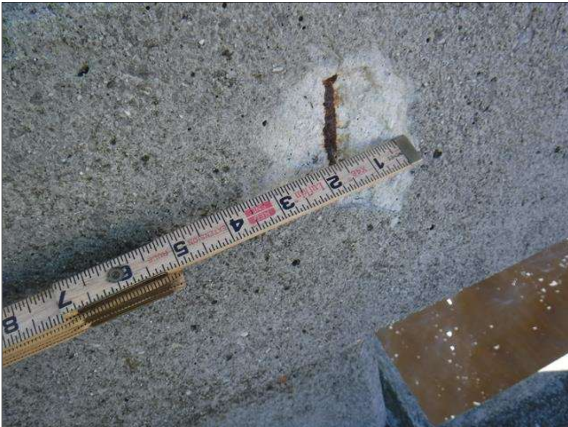
Span 47 Right Bridge Rail: 3" DIAMETER SPALL WITH EXPOSED REBAR ON LEFT FACE LOCATED AT POST 3 FROM BENT 46
