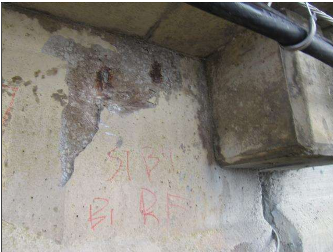
Span 1 Beam 4: 21" X 19" SURFACE SPALL WITH (2) UP TO 4" LONG EXPOSED REBARS, SOUTH FACE, 3' FROM BENT 1.
