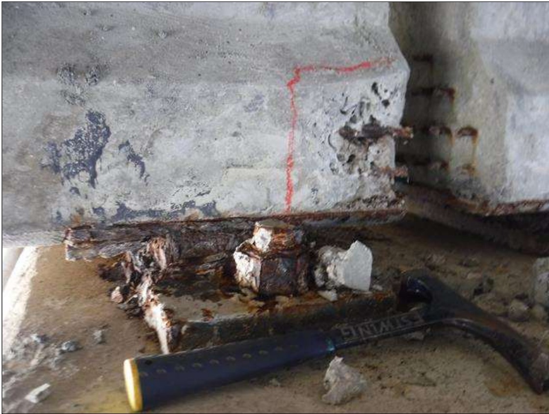
Span 207 Beam 3: (PAR) 6" X 6" X 2" DEEP SPALL WITH EXPOSED STRANDS IN BOTTOM FLANGE, NORTH FACE AT BENT 206
