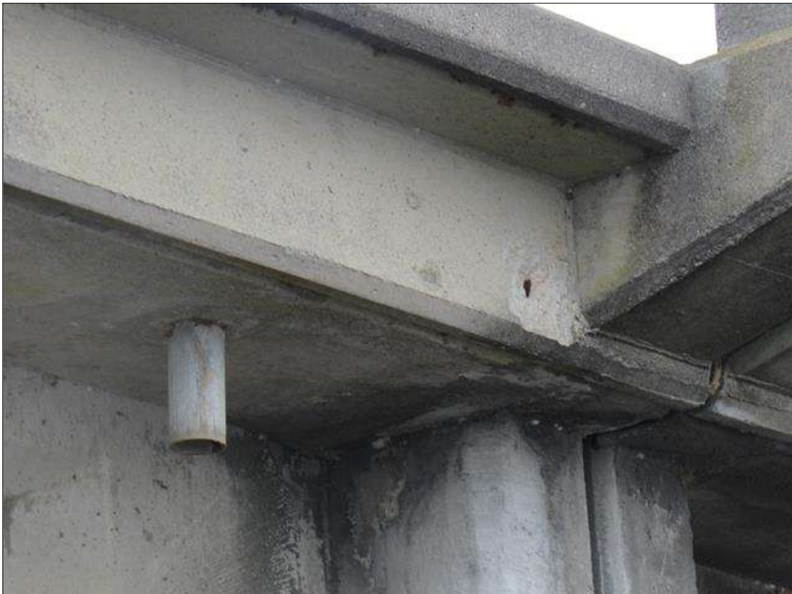
Span 267 Deck: 8" DIAMETER SPALL WTH EXPOSED REBAR ON UNDERSIDE OF DECK LOCATED ABOVE BENT
