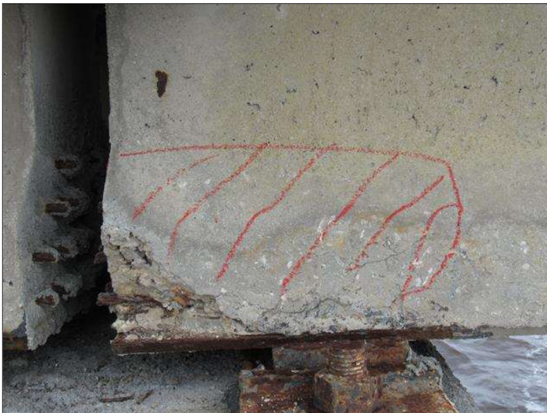
Span 48 Beam 4: (PAR) 9" X UP TO 5" X 2" DEEP SPALL WITH SURROUNDING DELAMINATION AND EXPOSED PRESTRESSING STRAND ON SOUTH FACE AT BENT 47
