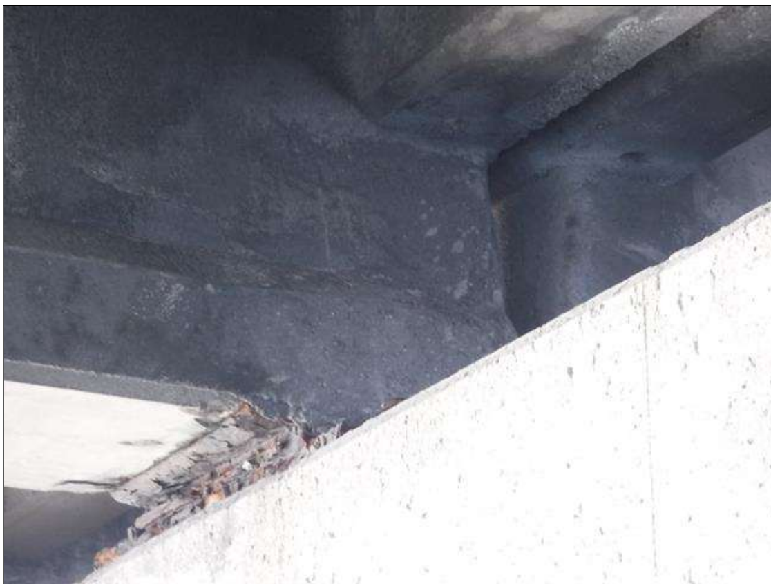
Span 16 Beam 3: (2) UP TO 18" X 12" PATCHED AREAS, NORTH AND SOUTH FACES, AT BENT 15.
