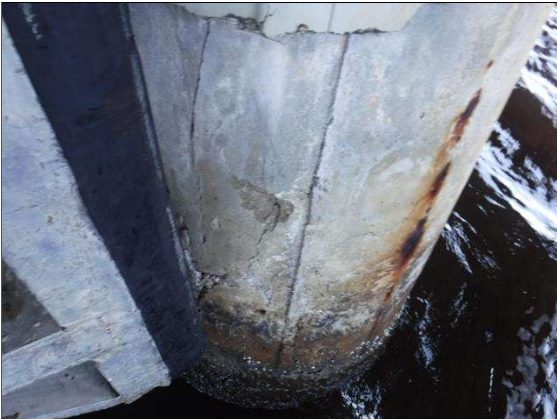
Bent 17 Saved Pile 2: JACKETED. SCALING TO 1" WITH LOOSE AGGREGATE FROM BOTTOM OF JACKET TO MUDLINE.
