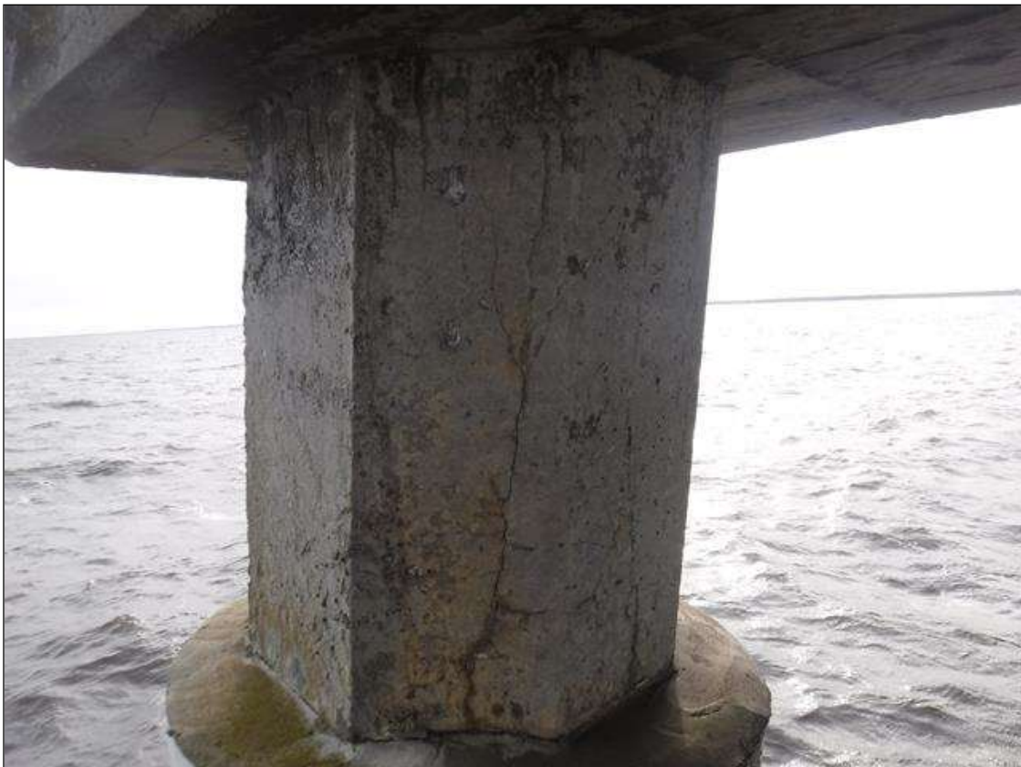
Bent 136 Saved Pile 4: 2' LONG X 0.006" VERTICAL CRACK ON EAST FACE
