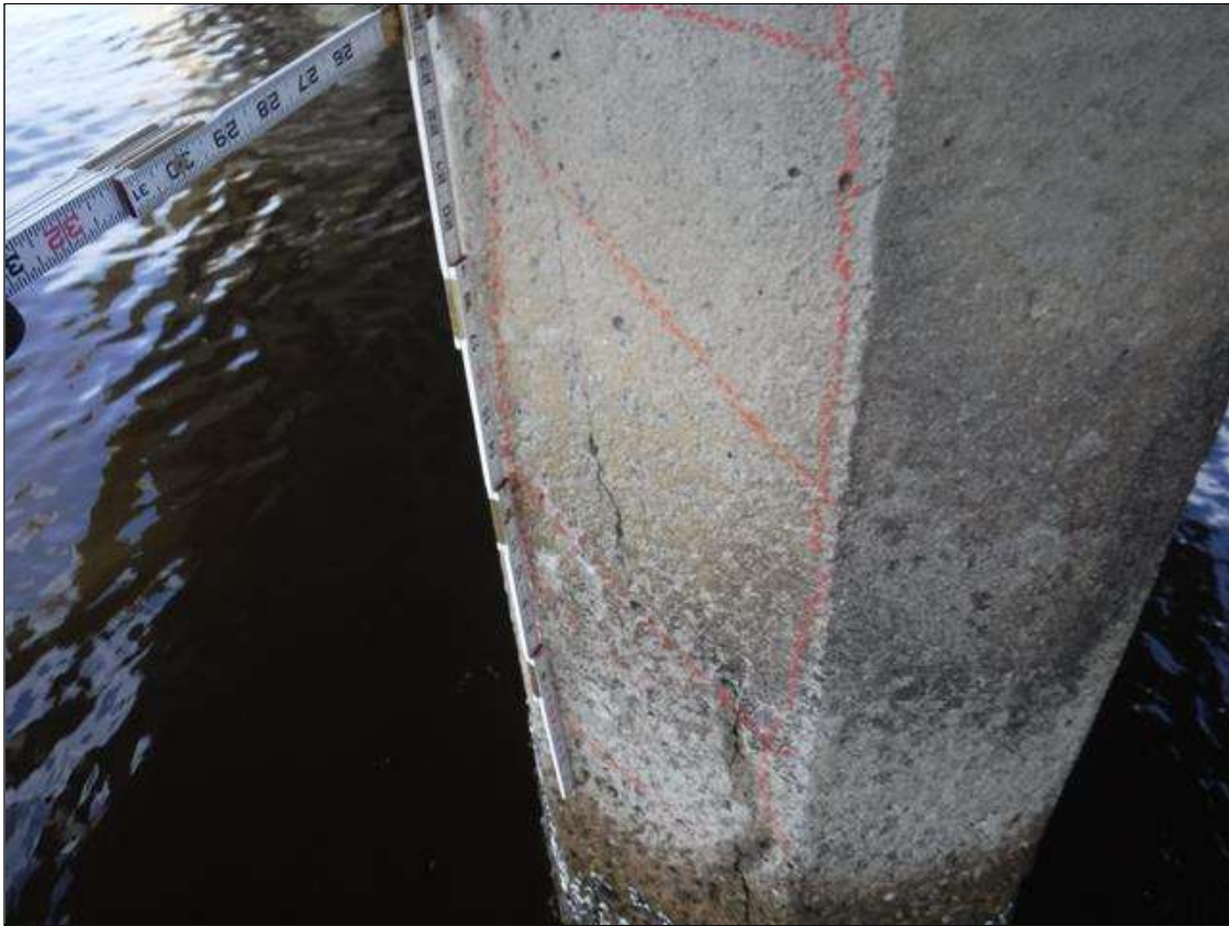
Bent 206 Pile 3: (PAR) HAIRLINE TO 1/16" CRACKS, 8' BELOW CAP, DOWN 4', MULTIPLE FACES. SCALING TO 1" DEEP WITH LOOSE AGGREGATE FROM WATERLINE TO MUDLINE.
