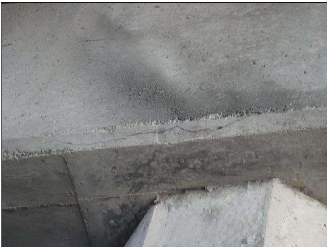
Bent 121 Cap 1: 12" X 2" DELAMINATION, BOTTOM FACE, WEST OF PILE 2.
