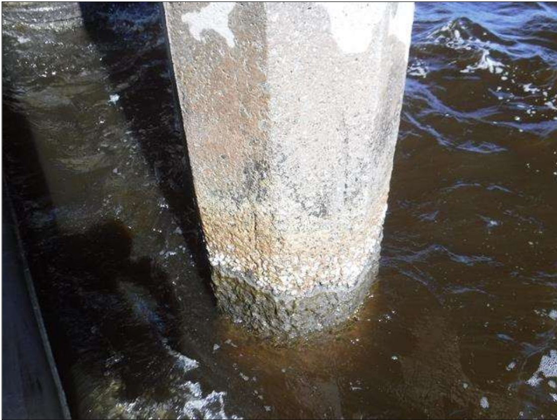
Bent 25 Saved Pile 6: 2' X 1' DELAMINATION, SOUTH FACE, 8' FROM BOTTOM OF CAP.
