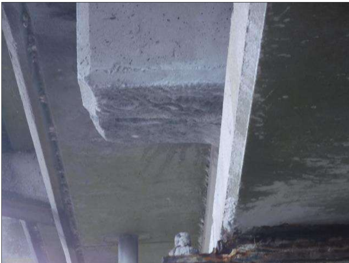
Span 156 Beam 1: 1' X UP TO 1' PATCHED AREA, END DIAPHRAGM, NORTH OVERHANG, AT BENT 155.
