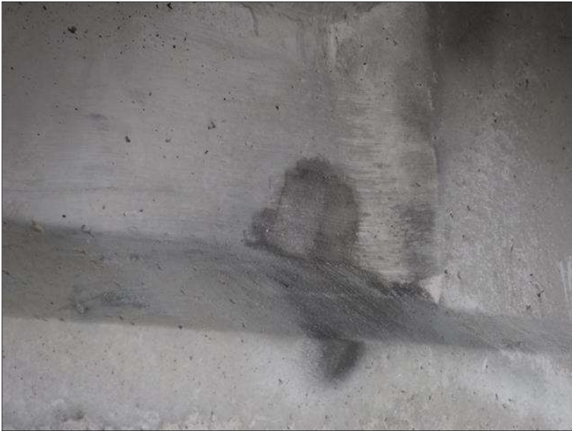
Span 204 Beam 2: 6" X 6" PATCHED AREA ON NORTH FACE IN WEB, 1' FROM BENT 203.
