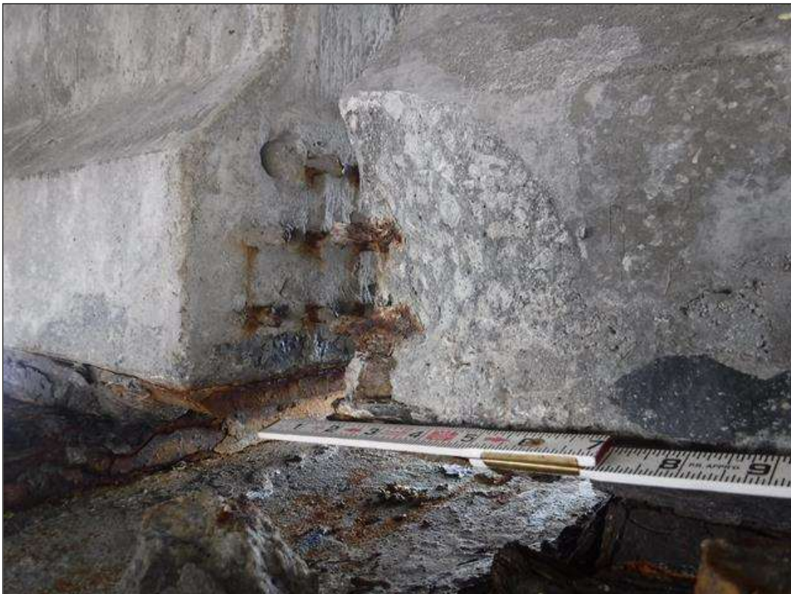
Span 205 Beam 1: (PAR) 6" X 6" X 2" DEEP SPALL WITH EXPOSED STRANDS IN BOTTOM FLANGE, SOUTH FACE AT BENT 204
