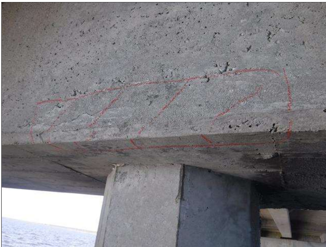
Bent 19 Cap 1: 48" X 12" X 12" CORNER FAILED PATCHED AREA, BOTTOM OF EAST FACE, BENEATH BEAM 2.
