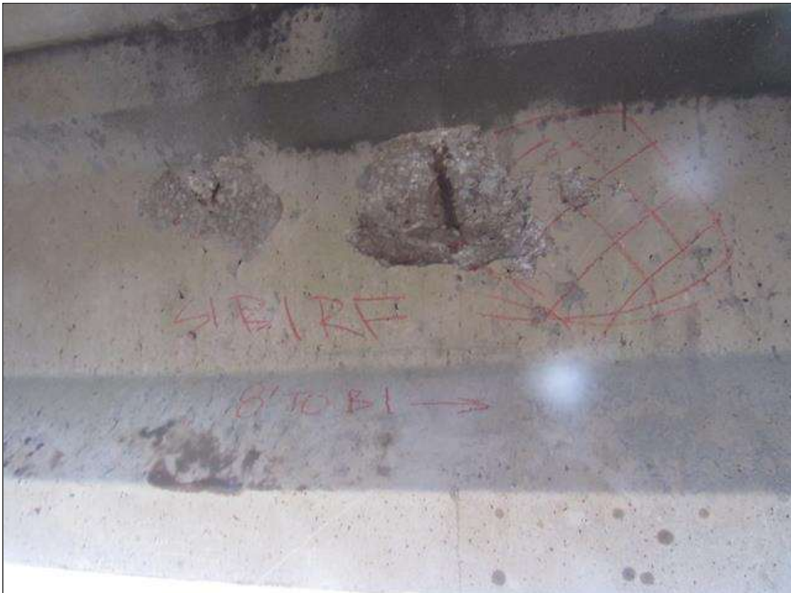
Span 1 Beam 1: (PAR) 4" X 6" X 2" SPALL, WITH EXPOSED STRAND, NORTH FACE, AT BENT 1.
