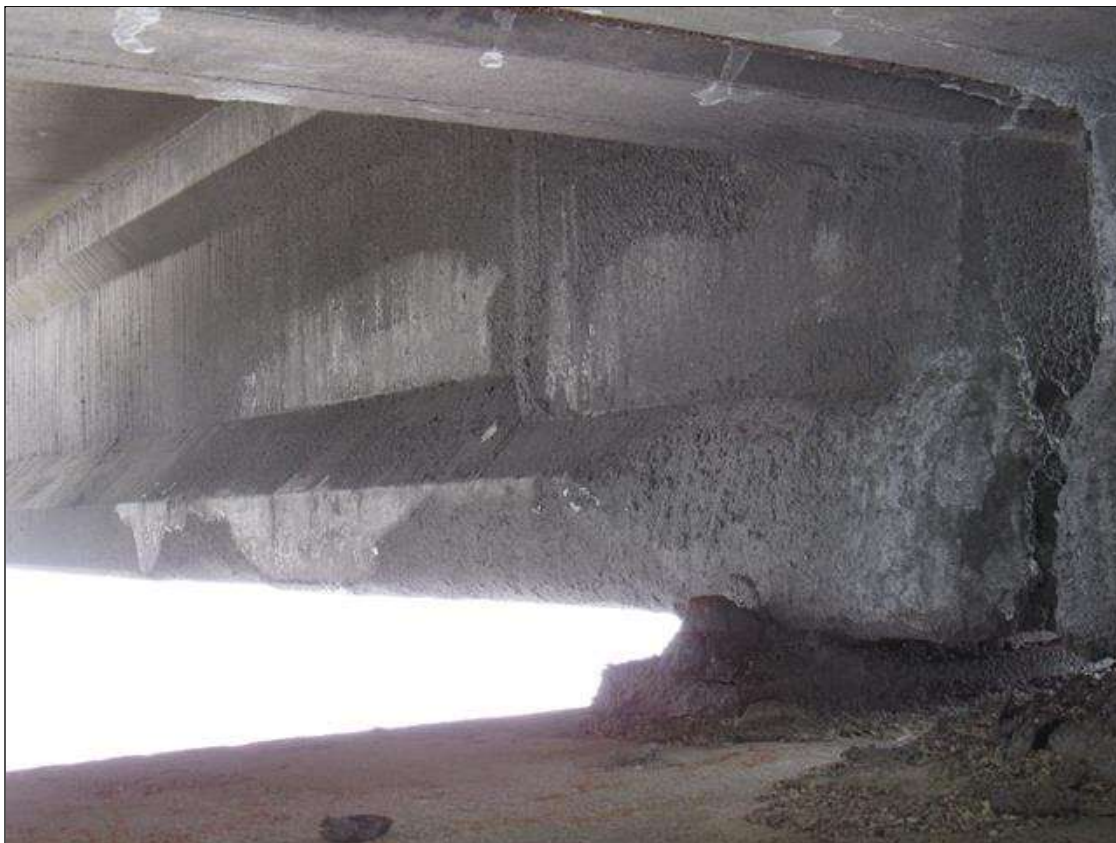
Span 47 Beam 4: 5' X UP TO 5" PATCHED AREA, BOTTOM FACE, EXTENDING 1' ONTO NORTH FACE, AT BENT 46.
