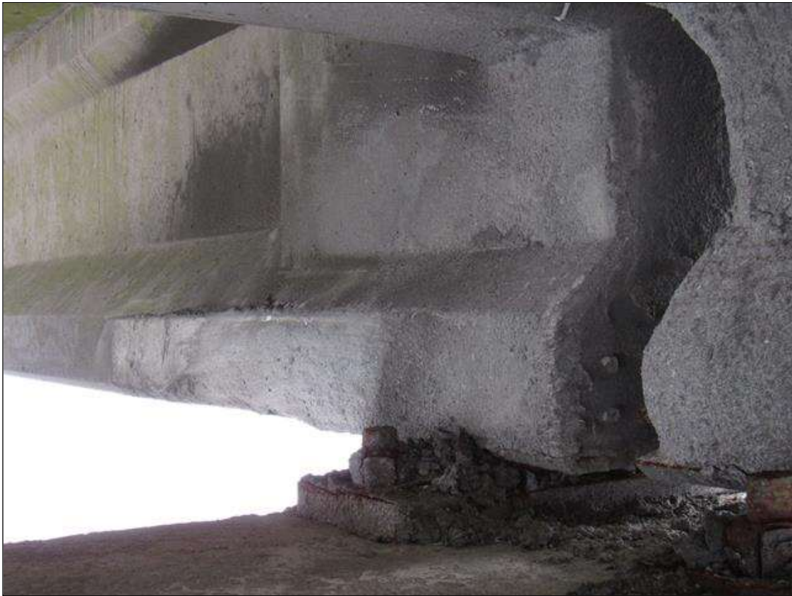
Span 52 Beam 4: 48" X 12" X 12" CORNER PATCHED AREA, NORTH FACE, AT BENT 51.
