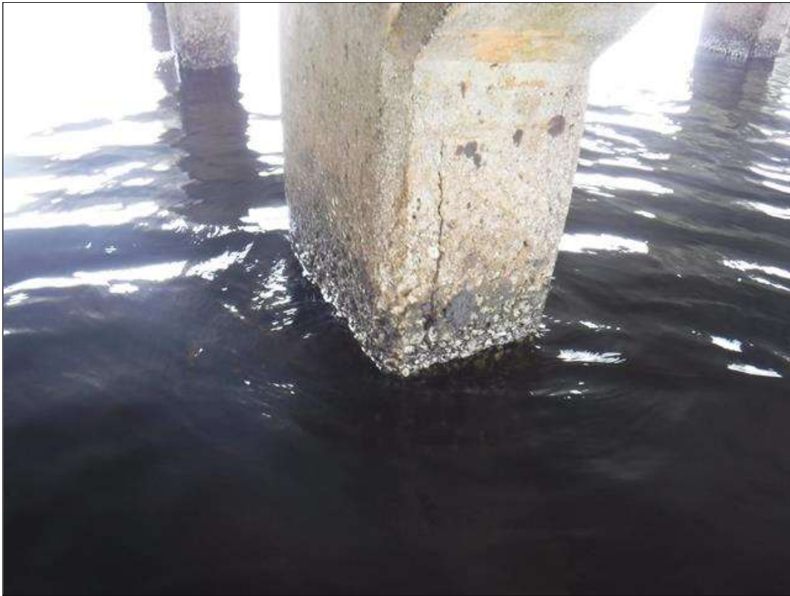
Bent 298 Pile 2: 16" X 2" DELAMINATION, NORTH FACE, AT BOTTOM OF CAP.
