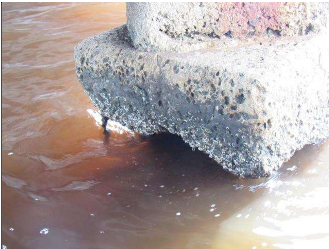
Bent 280 Pile 4: (PAR) 24" X 24" X 8" SPALL WITH EXPOSED REINFORCING ON EAST FACE
