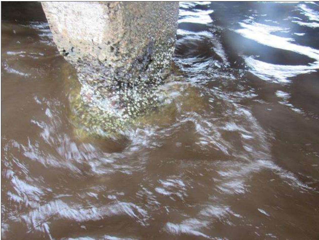
Bent 292 Pile 2: (PAR) SCALING AROUND BASE OF COLUMN AND TOP OF FOOTING 3" - 6" DEEP X 8" HIGH X 360*, EXPOSED REBAR WITH 25% SECTION LOSS.
