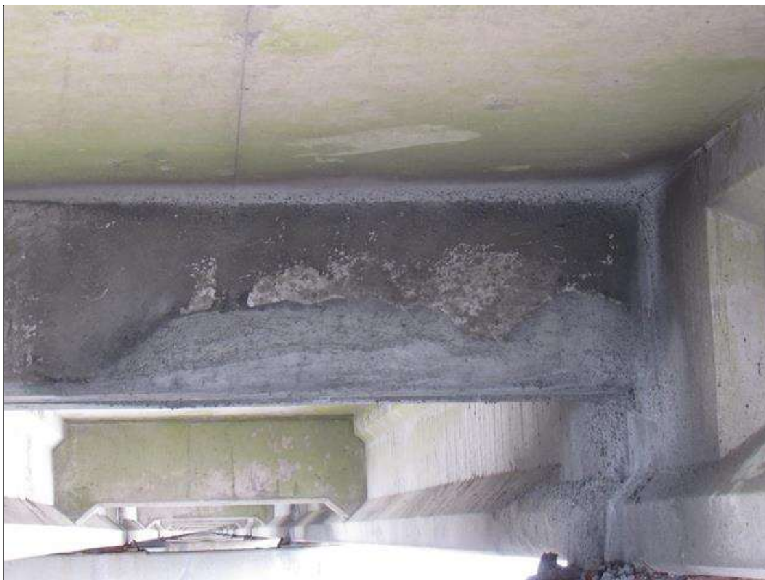
Span 47 Beam 3: 5' X UP TO 10" X 1' PATCHED AREA, WEST FACE, END DIAPHRAGM, BETWEEN BEAMS 3 AND 4, AT BENT 47.
