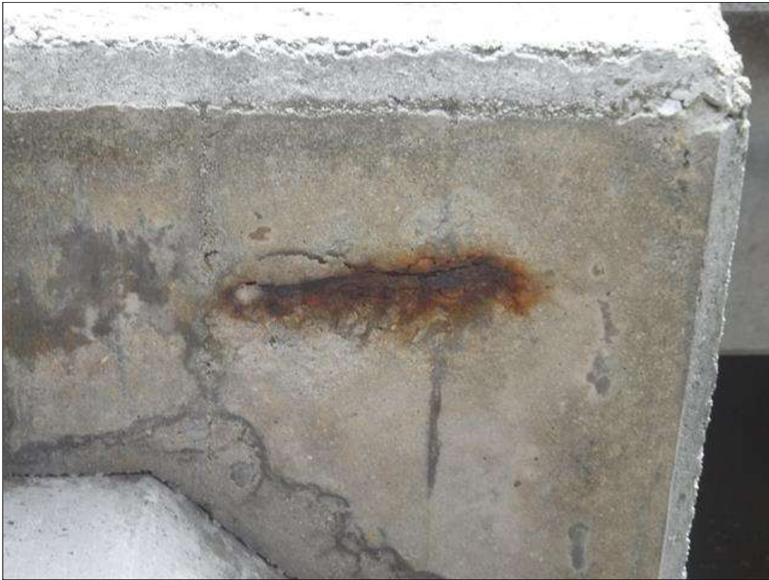
Bent 171 Cap 1: SPALL WITH EXPOSED REBAR IN BOTTOM OF RIGHT OVERHANG. AREA IS 4" LONG, 7" WIDE, AND 1.5" DEEP.
