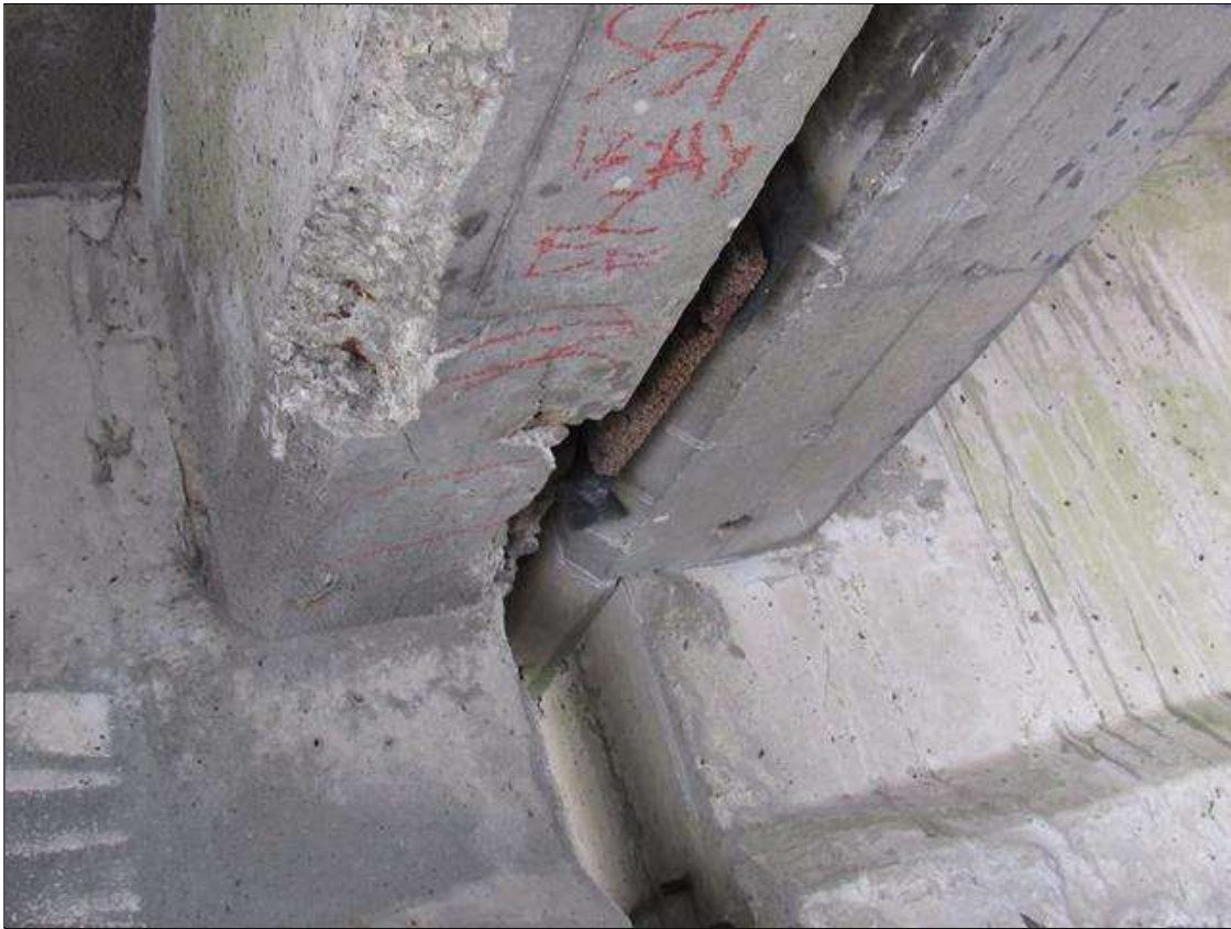
Span 51 Beam 2: 9" X UP TO 12" X 3" DEEP SPALL WITH SURROUNDING DELAMINATION AT BOTTOM WEST CORNER OF END DIAPHRAGM IN BAY 2 AT BENT 50
