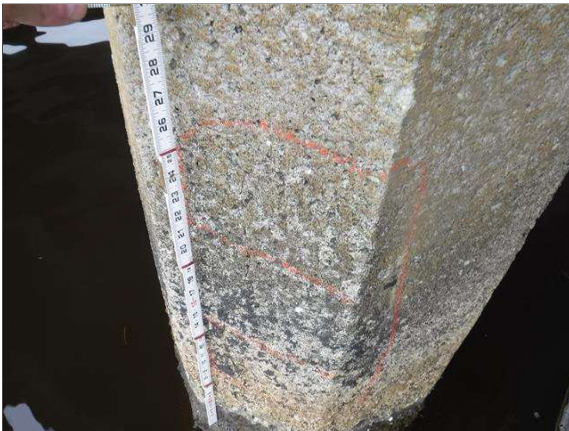
Bent 244 Pile 1: (PAR) (2) UP TO 3' X 0.03" VERTICAL CRACKS WITH 2' X 1' SURROUNDING DELAMINATION ON NORTH FACE, BEGINNING 7' FROM BOTTOM OF CAP, AT RANDOM THROUGHOUT.
