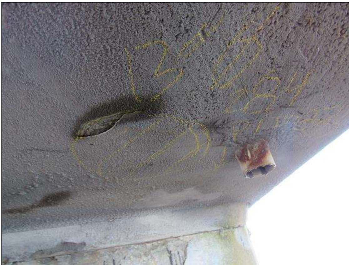
Span 284 Deck: 13" DIAMETER DELAMINATION ON BOTTOM FACE LOCATED NEAR BENT 283 PILE 1
