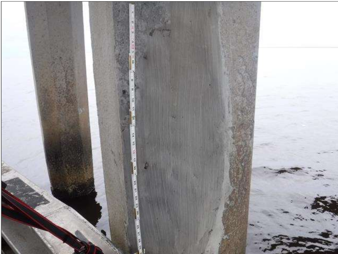
Bent 252 Pile 3: 4' X 14" PATCHED AREA ON NORTH FACE, BEGINNING 4' FROM BOTTOM OF CAP.
