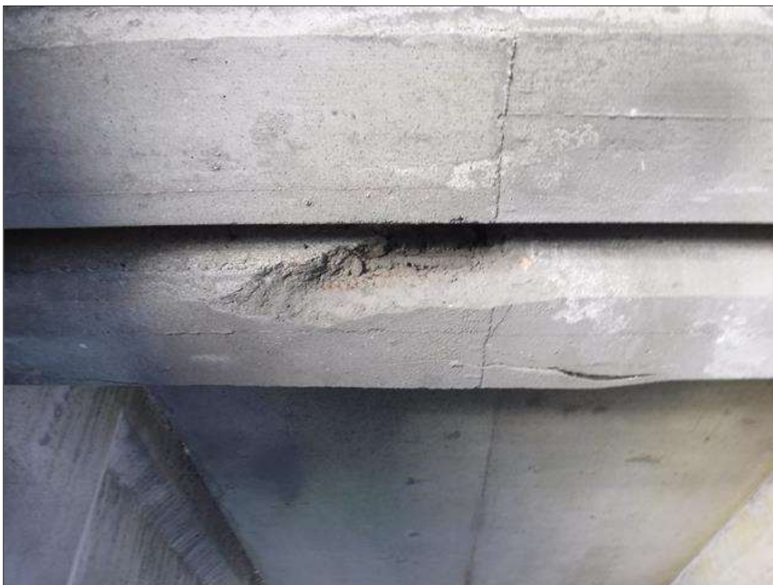
Span 13 Beam 1: 18" X 6" X 3" DEEP SPALL IN BENT 13 DIAPHRAGM
