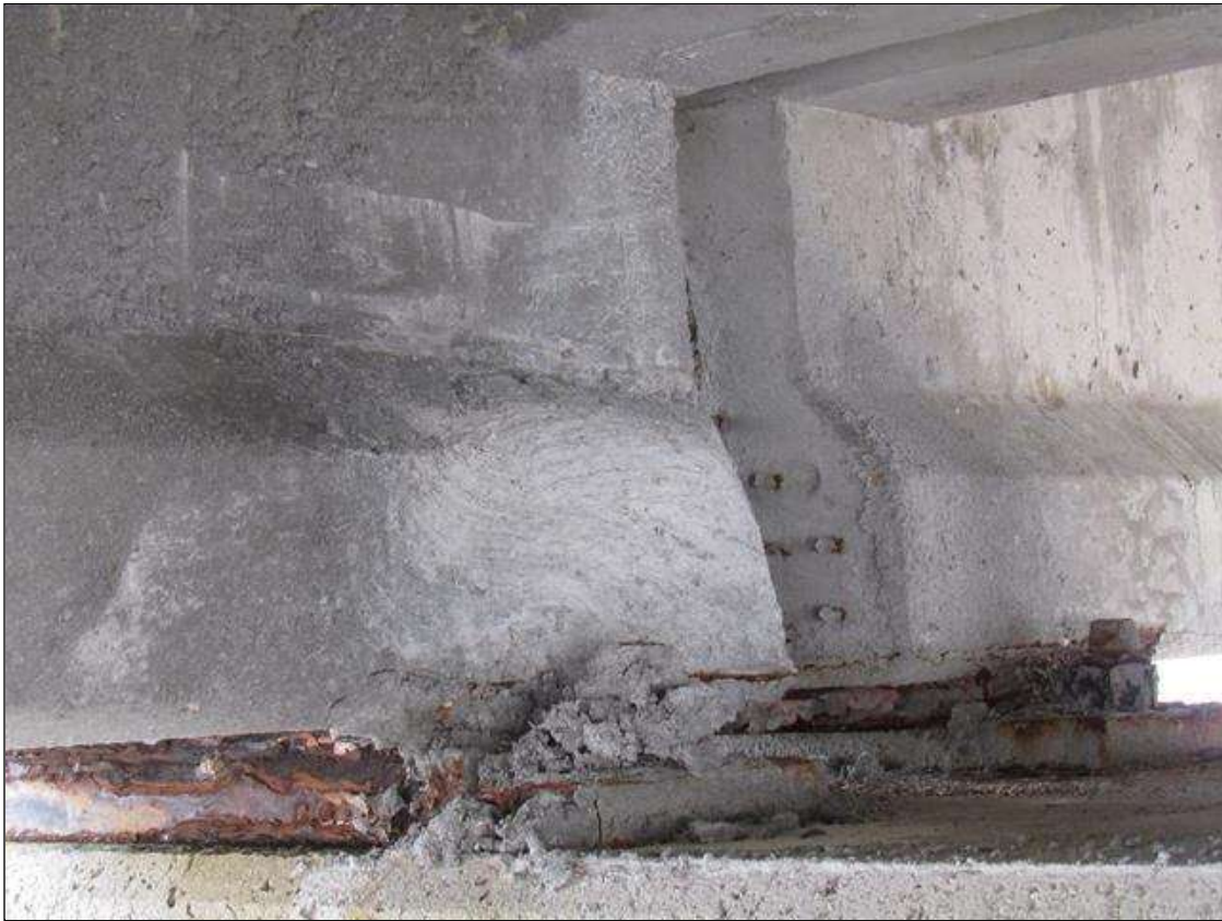
Span 65 Beam 1: 18" X 12" PATCHED AREA, SOUTH FACE, AT BENT 65.
