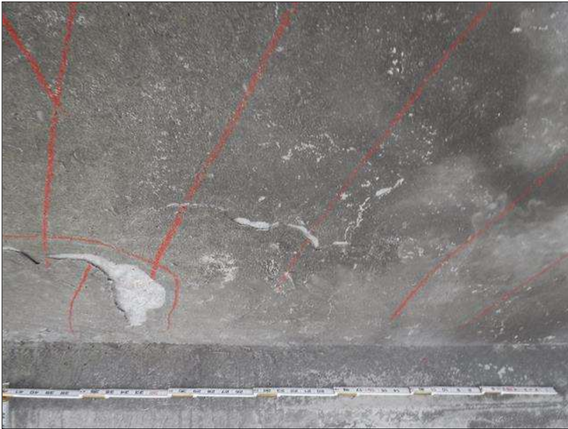
Span 232 Deck: (PAR) 6' X 4' AREA OF DELAMINATION, DECK UNDERSIDE, BETWEEN BEAMS 1 AND 2, NEAR BENT 231.
