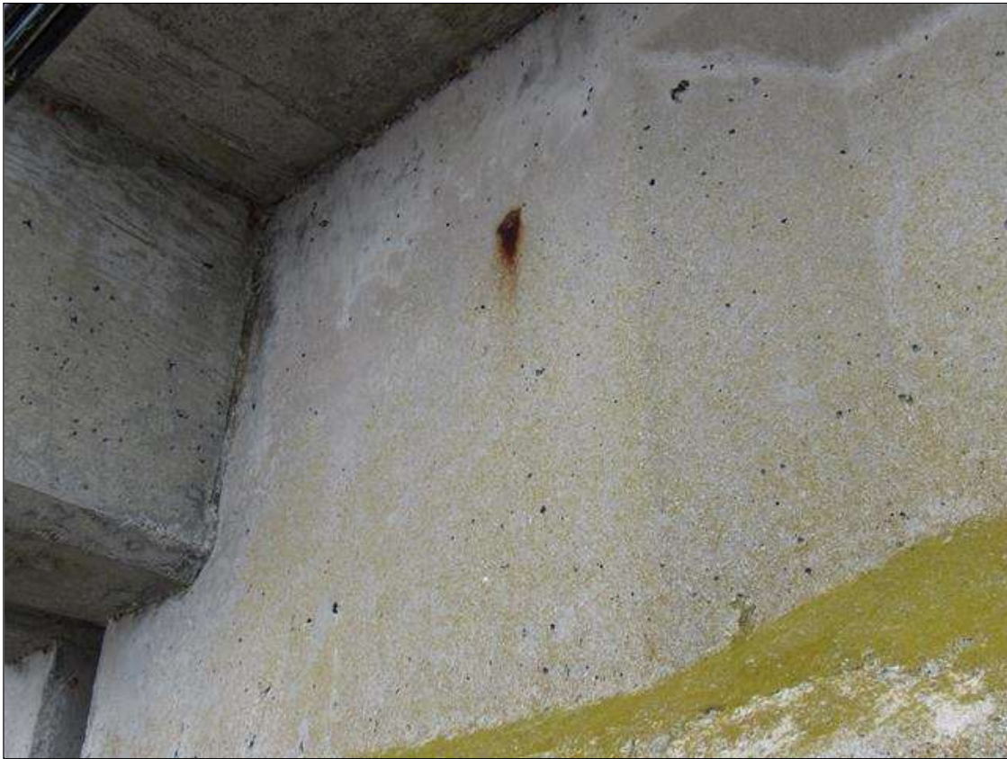
Span 51 Beam 1: 1" X 2" AREA OF RUST STAINING, NORTH FACE, 1' FROM BENT 51.
