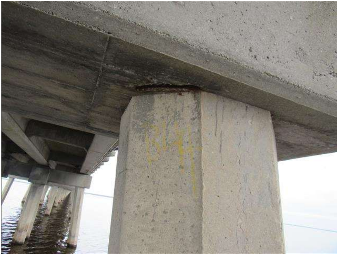
Bent 44 Cap 1: 8" X 1.5" X 3/4" DEEP SPALL WITH EXPOSED REINFORCING ON BOTTOM WEST CORNER LOCATED AT TOP OF PILE 4
