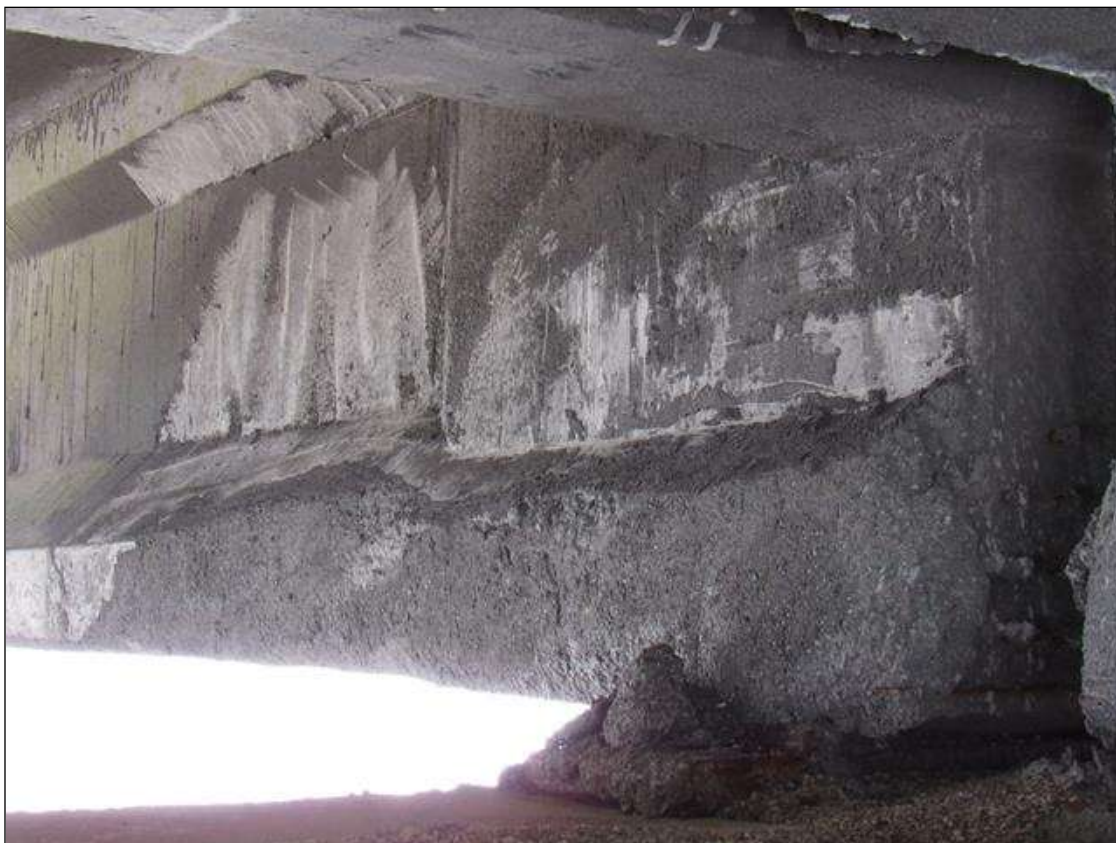
Span 44 Beam 2: 5' X UP TO 10" PATCHED AREA, BOTTOM FACE, EXTENDING 6" ONTO NORTH FACE, AT BENT 43.
