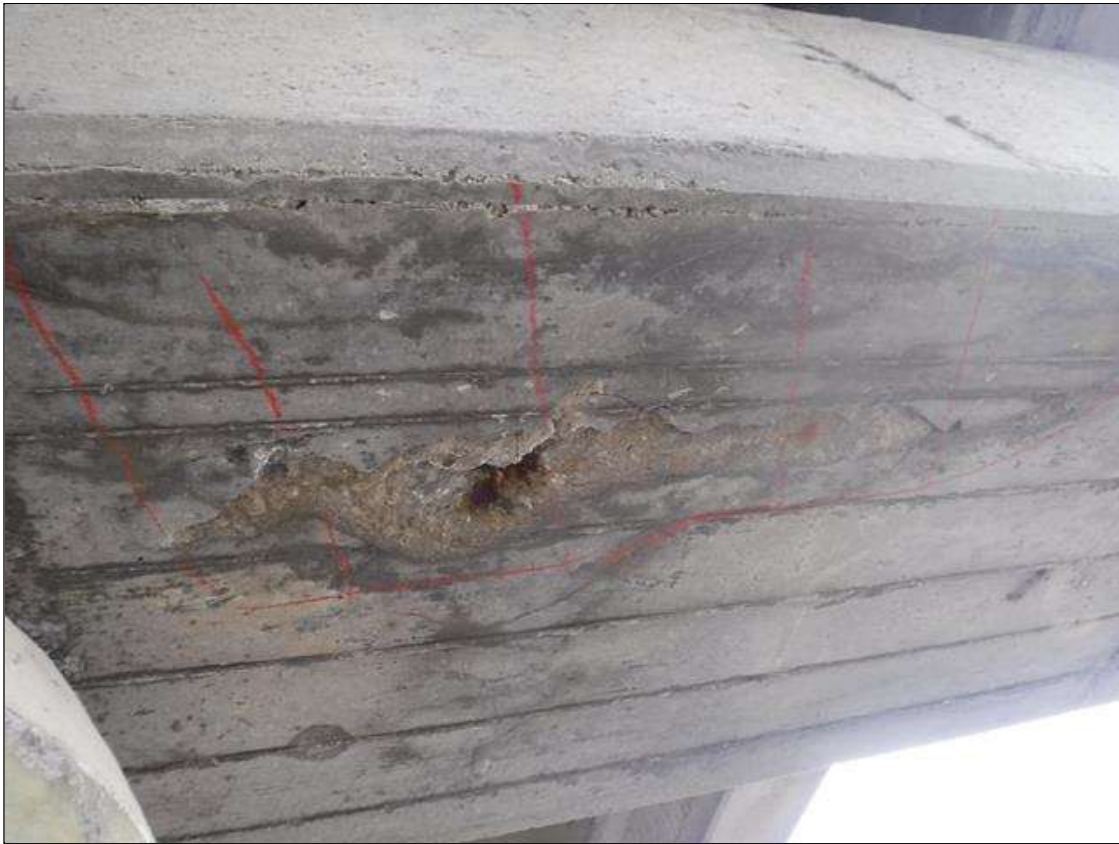
Bent 238 Cap 1: 12" X 6" X 1" SPALL WITH EXPOSED REINFORCING WITH 4' X 18" OF SURROUNDING DELAMINATION ON BOTTOM FACE, BETWEEN BEAMS 1 AND 2.
