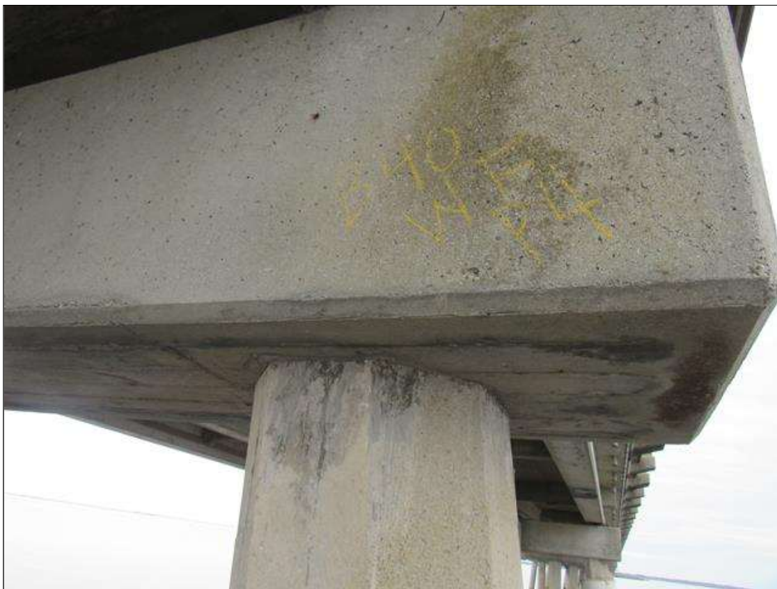
Bent 40 Cap 1: 3' X 14" DELAMINATION, BOTTOM OF CAP, AT PILE 4, EXTENDING 6" ONTO WEST FACE. NOT OBSERVED IN 2020 INSPECTION
