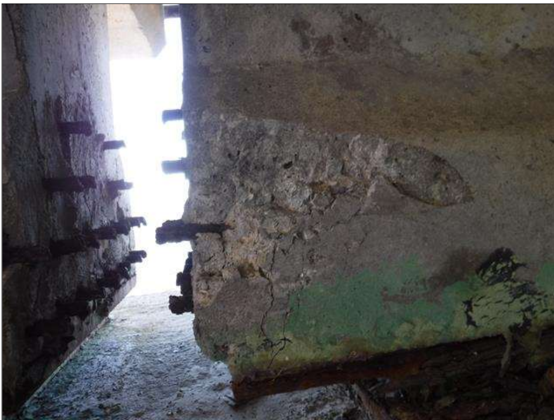
Span 9 Beam 4: (PAR) 6" X 4" X 2" SPALL, WITH EXPOSED STRAND, NORTH FACE, AT BENT 9.
