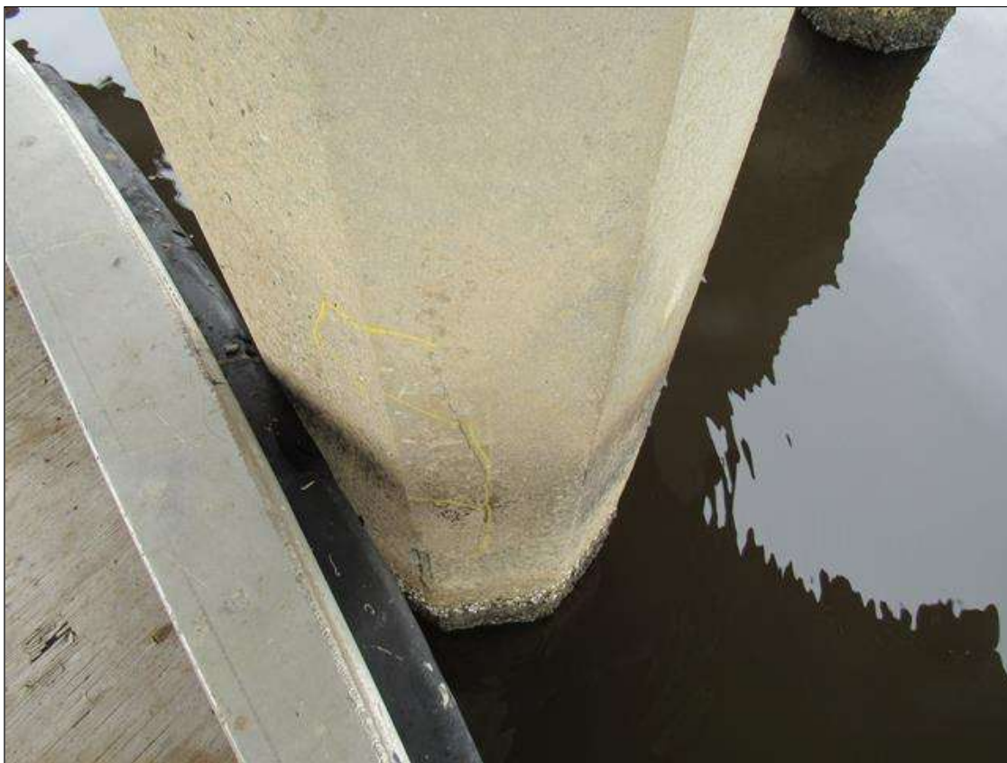
Bent 31 Saved Pile 2: 1' X 3' DELAMINATION ON SOUTH FACE LOCATED 7' FROM BOTTOM OF CAP
