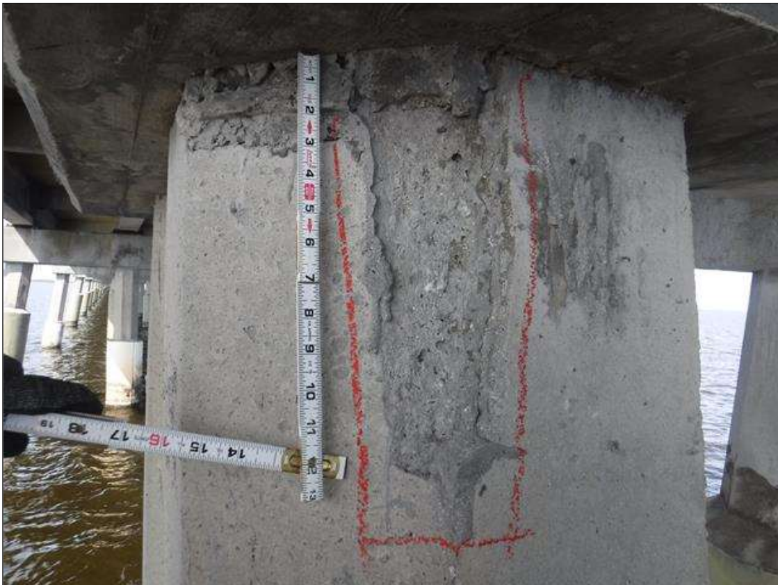
Bent 223 Pile 5: 12" X UP TO 4" X 1/2" SPALL, EAST FACE, AT BOTTOM OF CAP.
