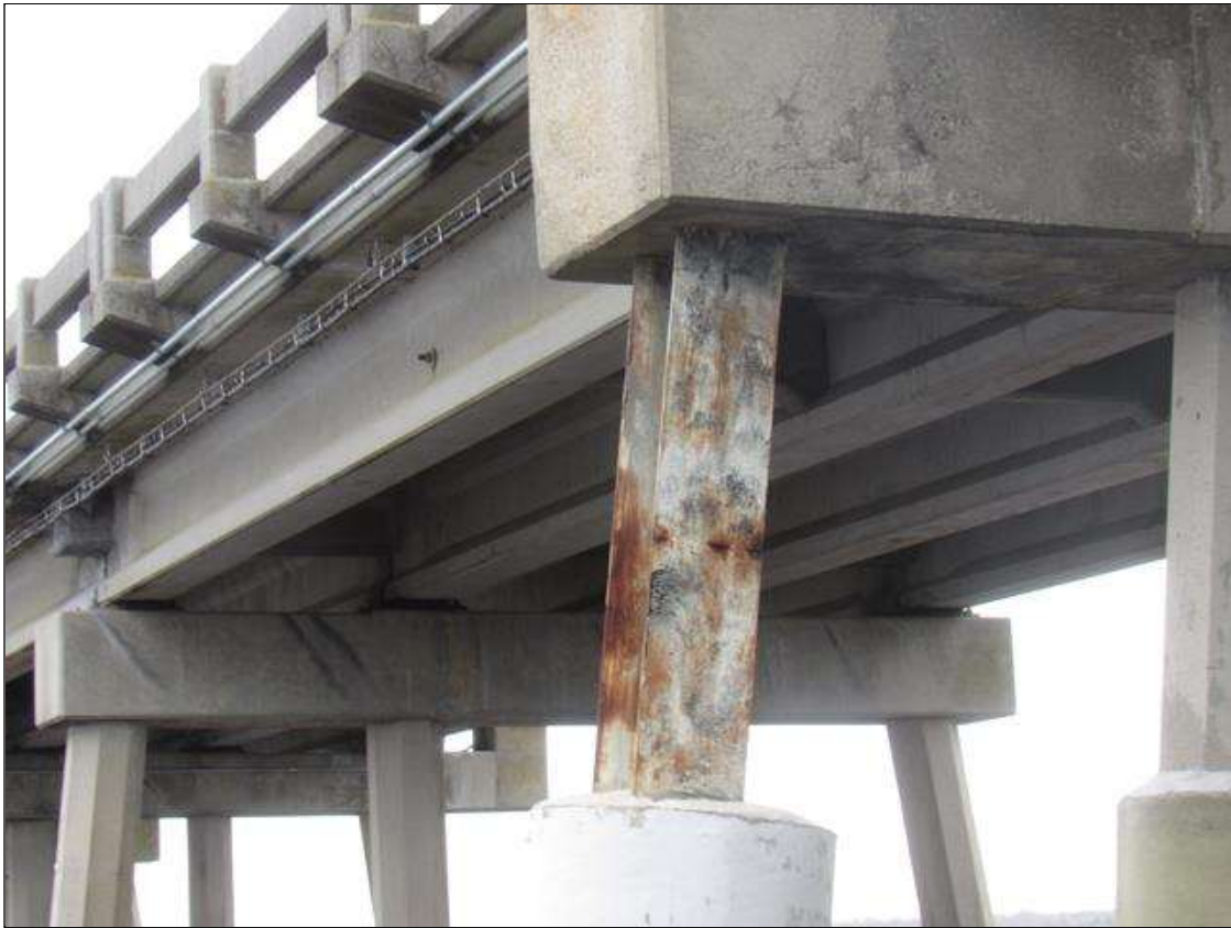
Bent 112 Pile 5: 4' SURFACE RUST, AT RANDOM THROUGHOUT.
