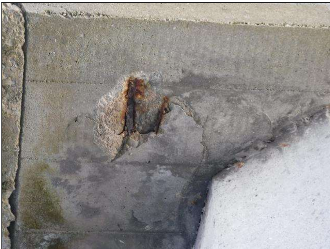
Bent 120 Cap 1: 8" DIAMETER X 1/2" SPALL, WITH EXPOSED REINFORCING, BOTTOM FACE, NEAR PILE 2.
