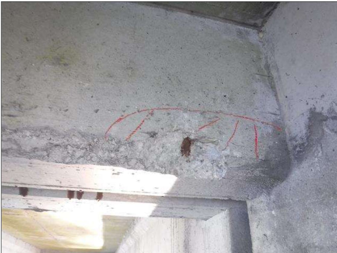
Span 126 Beam 2: 6" DIAMETER X 2" DEEP SPALL WITH 1' DELAMINATION, WEST FACE OF BENT 126 DIAPHRAGM, BETWEEN BEAMS 2 AND 3.
