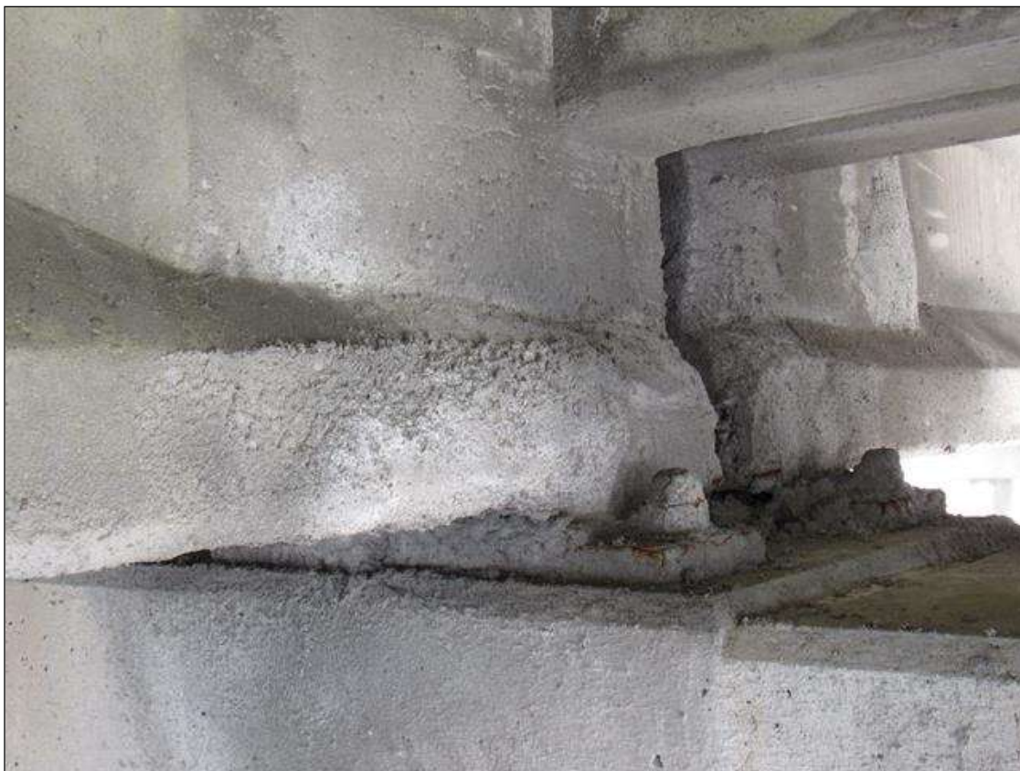
Span 60 Beam 3: (2) UP TO 24" X 12" X 4" CORNER PATCHED AREAS, NORTH AND SOUTH FACES, AT BENT 60.
