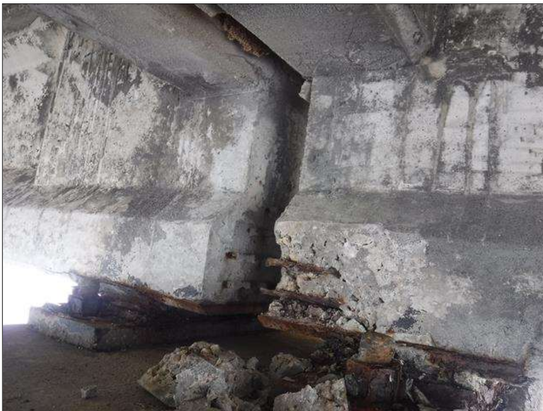
Span 98 Beam 3: (PAR) 6" X 6" X 2" DEEP SPALL WITH EXPOSED STRAND ON SOUTH FACE AT BENT 98
