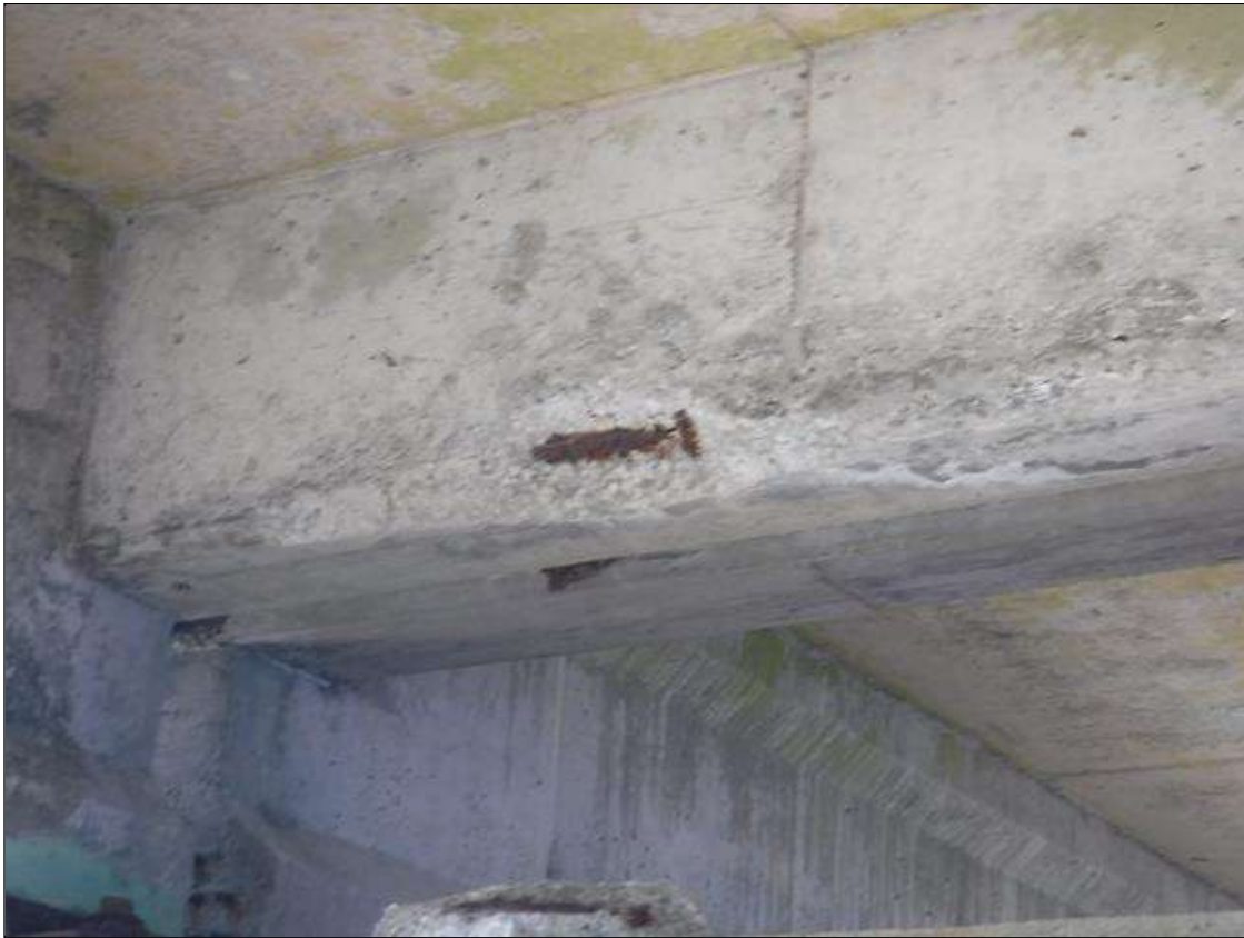
Span 23 Beam 4: 2' X 10" X 1" DEEP SPALL WITH EXPOSED REBAR ON BENT 22 DIAPHRAGM
