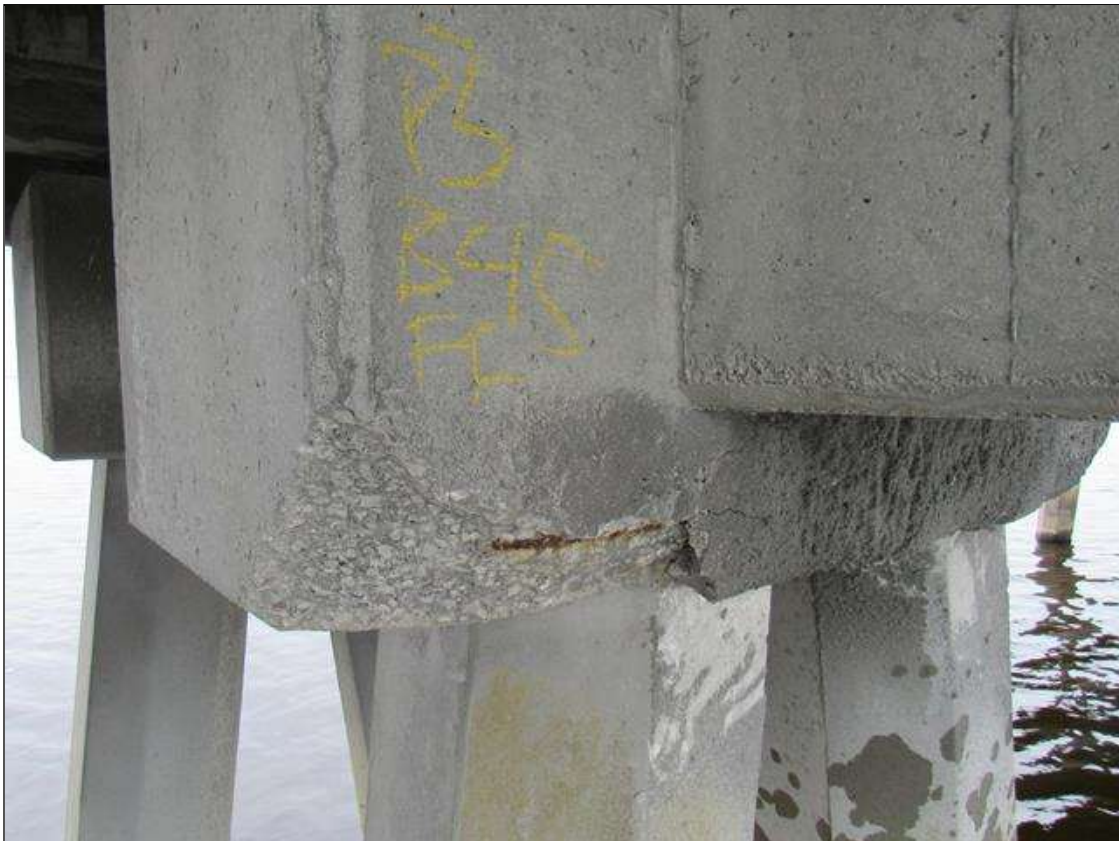
Bent 45 Cap 1: (PAR) 17" X 8" X UP TO 11" DEEP SPALL WITH 9" OF EXPOSED REBAR ON EAST FACE LOCATED LEFT OF PILE 3. REBAR HAS 10% SECTION LOSS
