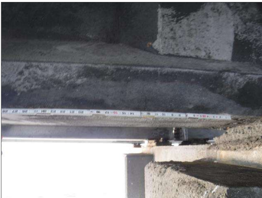
Span 10 Beam 2: (2) UP TO 24" X 6" X 12" CORNER PATCHED AREAS, NORTH AND SOUTH FACES, AT BENT 9.
