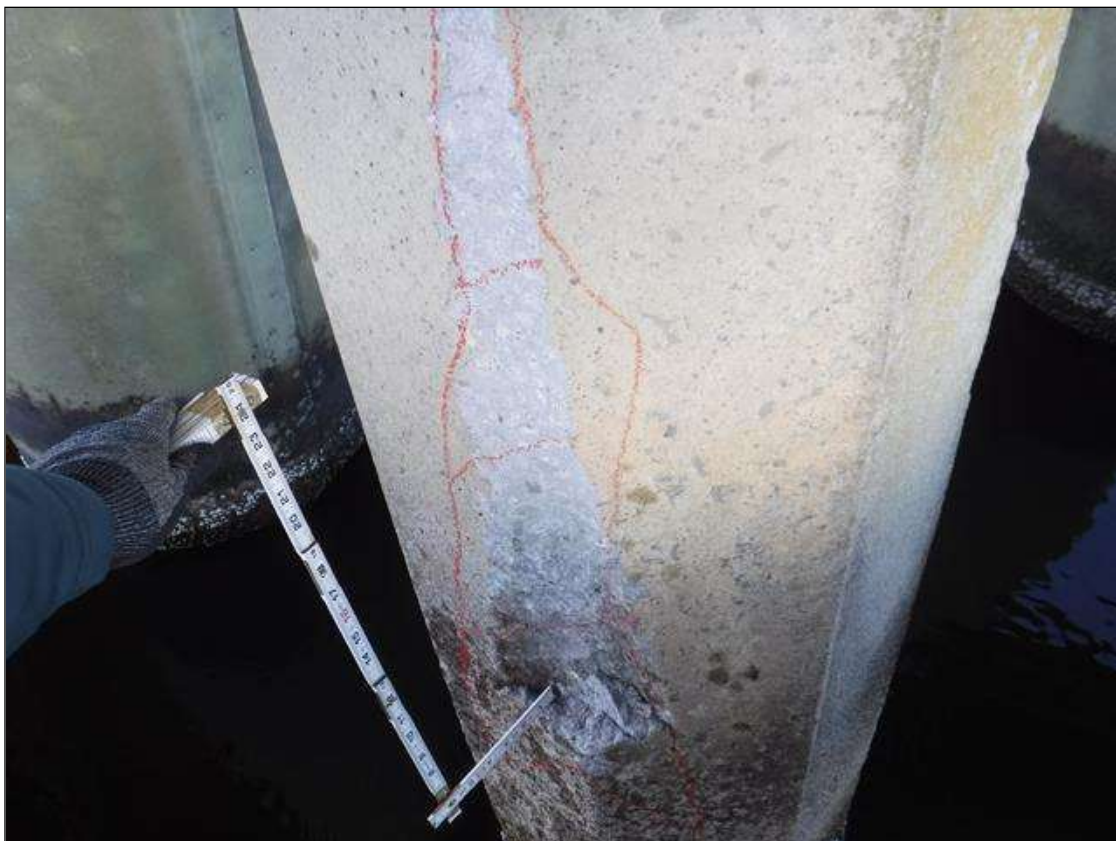
Bent 211 Pile 5: (PAR) 4' HIGH X 16" WIDE X 2" DEEP SPALL ON SOUTH FACE 8' BELOW CAP
