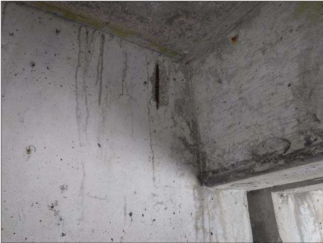
Span 86 Beam 2: 9" X 2" X 1/2" DEEP SPALL WITH EXPOSED REBAR ON SOUTH FACE IN WEB AT BENT 86
