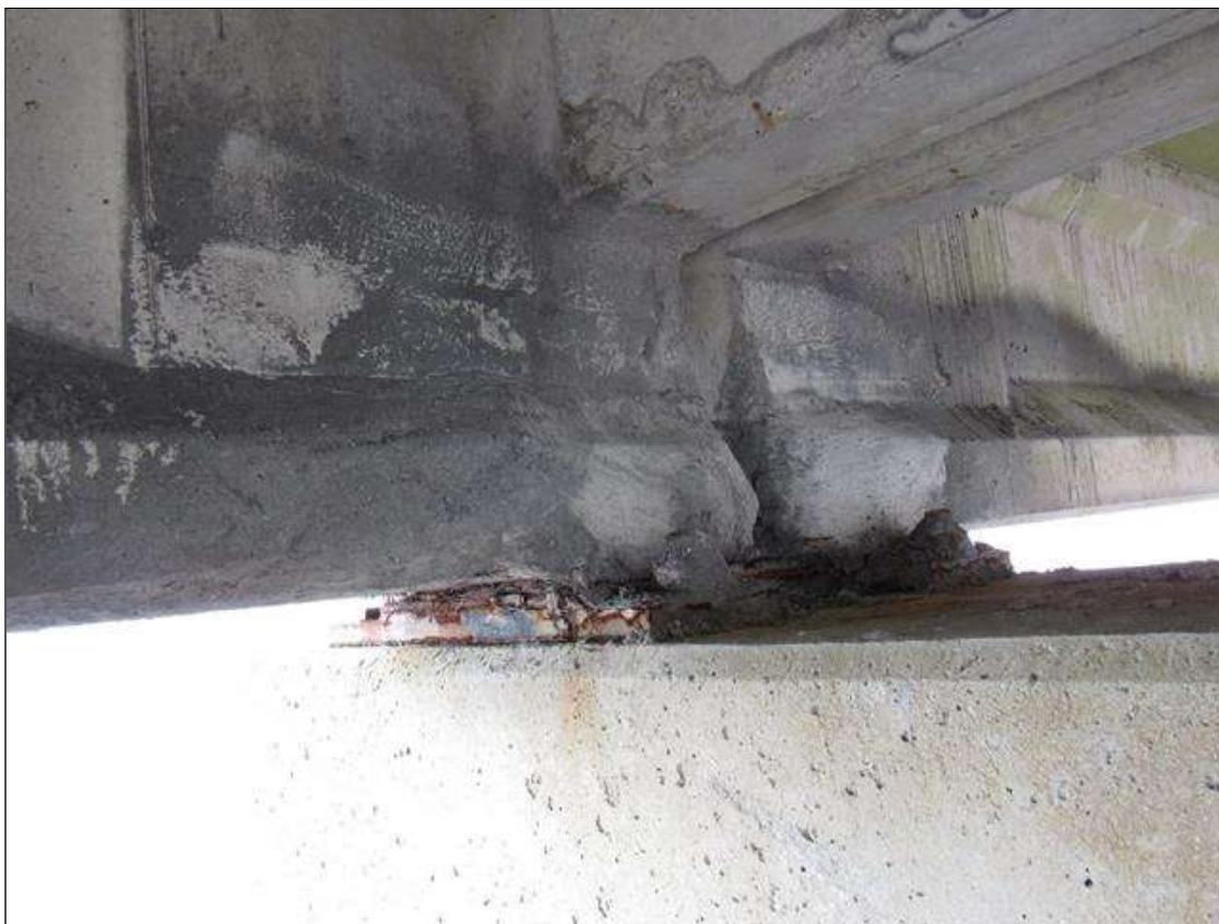
Span 56 Beam 1: 48" X 18" X 6" CORNER PATCHED AREA, SOUTH FACE, AT BENT 56.
