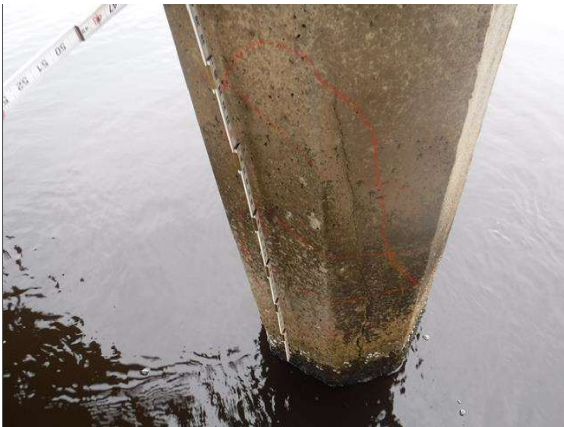
Bent 242 Pile 1: (PAR) HAIRLINE TO 1/8" CRACKS, 8' BELOW CAP, DOWN 4' , MULTIPLE FACES. SCALING TO 1" DEEP WITH LOOSE AGGREGATE FROM WATERLINE TO MUDLINE.
