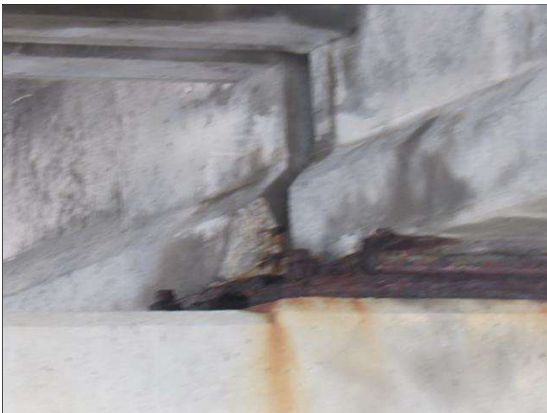
Span 274 Beam 2: (PAR) 6" X 6" X 1" SPALL, WITH EXPOSED STRAND, NORTH FACE, AT BENT 273.
