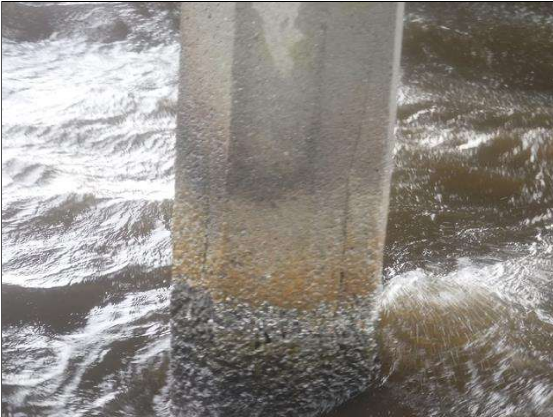
Bent 88 Pile 2: (PAR) UP TO 3' X 0.06" VERTICAL CRACK WITH SURROUNDING 4' X 2' DELAMINATION ON WEST FACE, BEGINNING 8' BOTTOM OF CAP, AT RANDOM THROUGHOUT.
