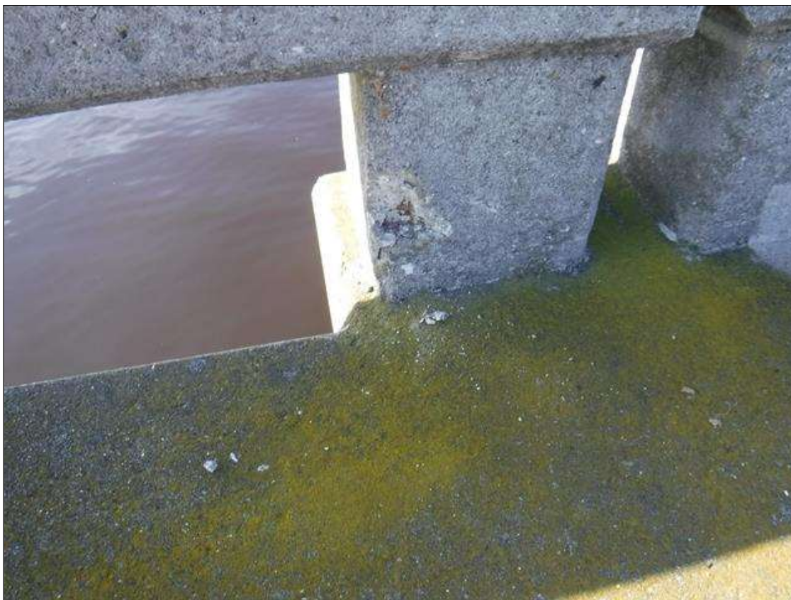
Span 265 Right Bridge Rail: 8" X 3" X 3" SPALL WITH EXPOSED REBAR AT BOTTOM LEFT CORNER LOCATED ON POST 4
