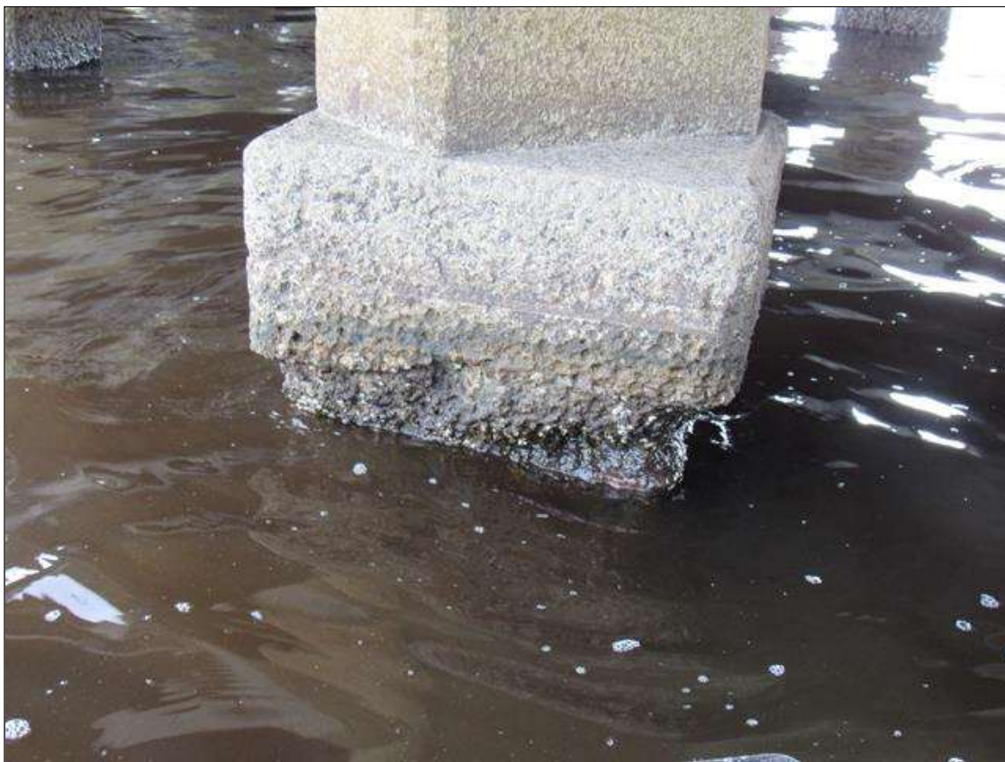
Bent 278 Pile 1: (PAR) 8' X 1' X 8" DEEP SPALL WITH EXPOSED REINFORCING LOCATED ON ALL FACES
