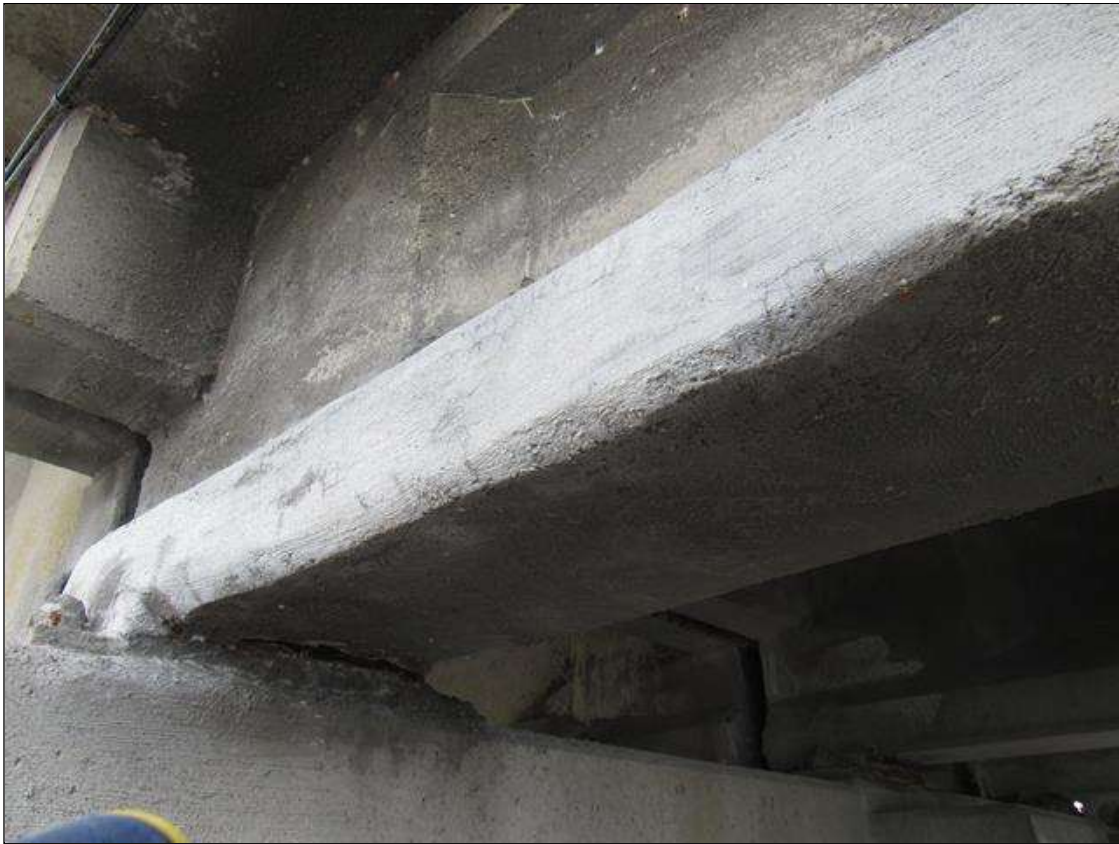
Span 33 Beam 1: 4' X 1' PATCHED AREA, NORTH FACE, AT BENT 33.
