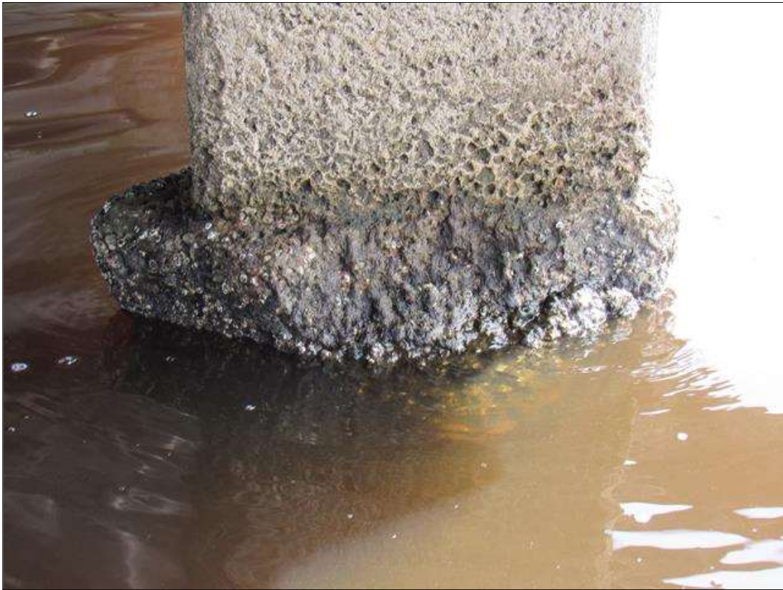
Bent 284 Pile 4: (PAR) 18" X 24" X 24" SPALL, WITH EXPOSED REBAR WITH COMPLETE SECTION LOSS TO VERTICAL BARS, WEST FACE OF COLUMN FOOTING.
