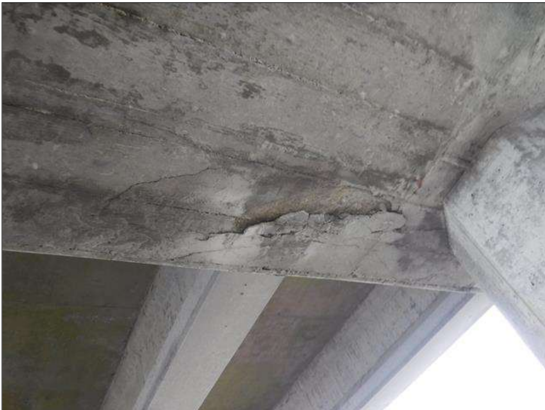
Bent 186 Cap 1: 3' OF DELAMINATION IN BOTTOM OF CAP ON EAST SIDE AT PILE 3.
