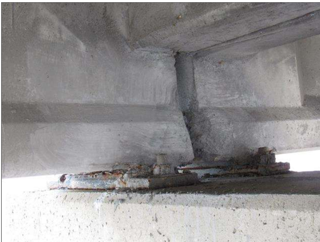
Span 66 Beam 1: 9" X 8" PATCHED AREA, SOUTH FACE, AT BENT 66.
