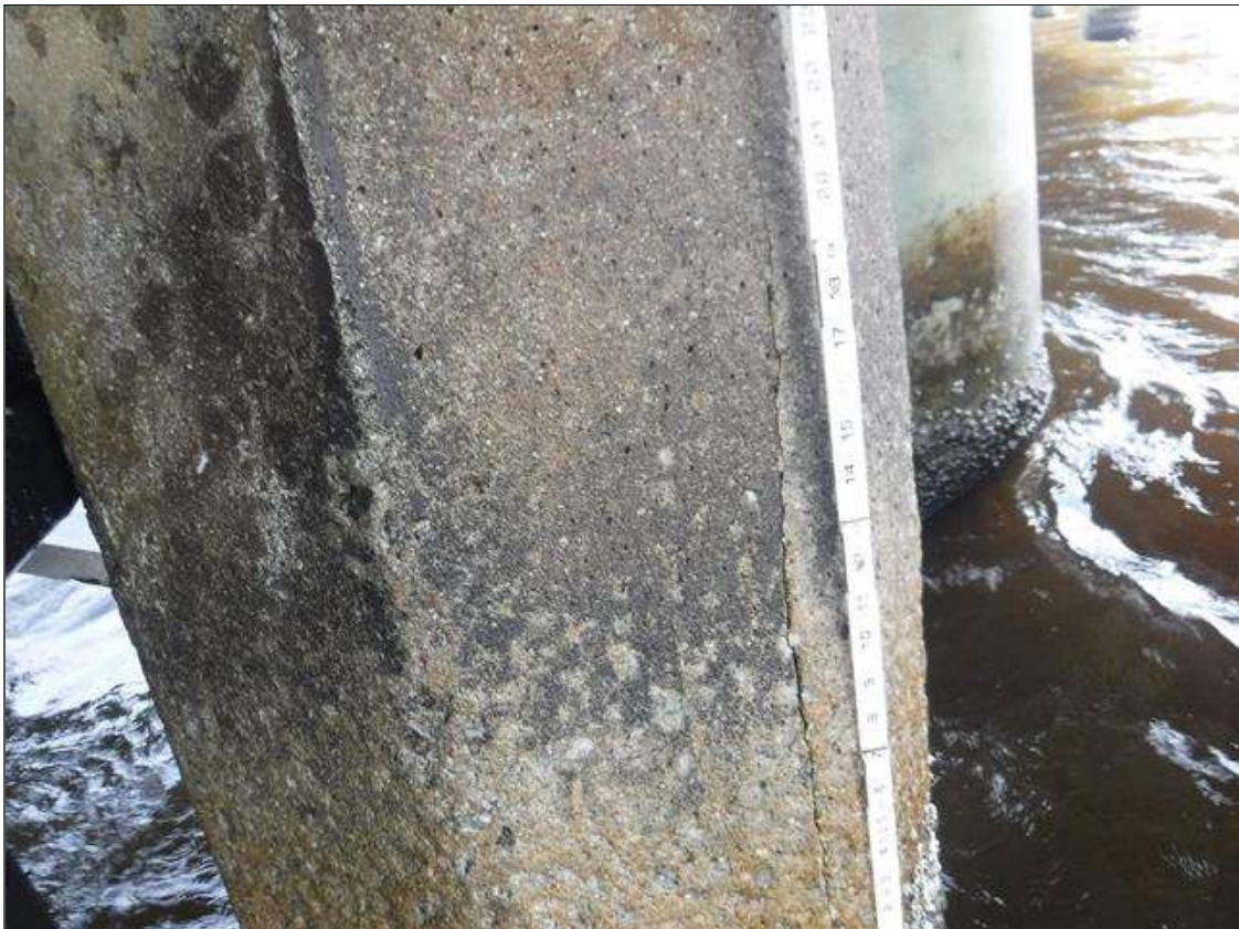
Bent 171 Pile 2: (PAR) 3' X 0.03" VERTICAL CRACK, WEST FACE, BEGINNING 7' FROM BOTTOM OF CAP.
