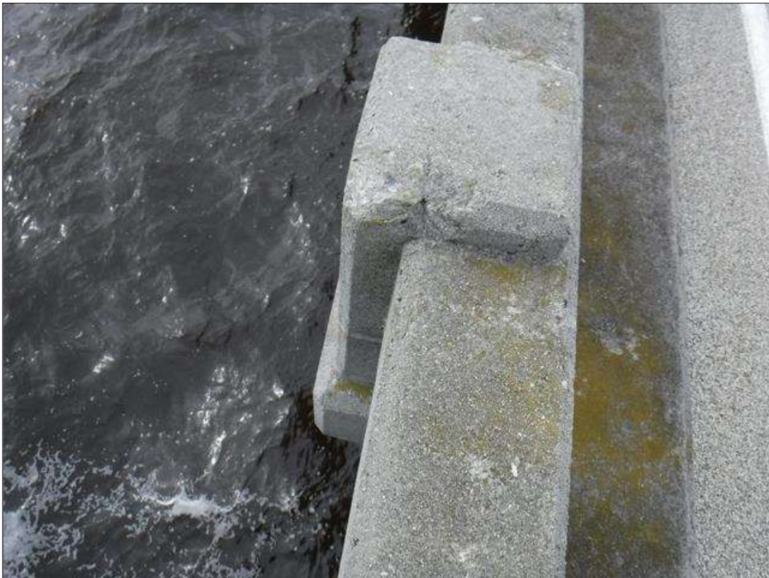
Span 218 Right Bridge Rail: 6" X 3" X 3" SPALL AT TOP RIGHT CORNER LOCATED ON POST 5
