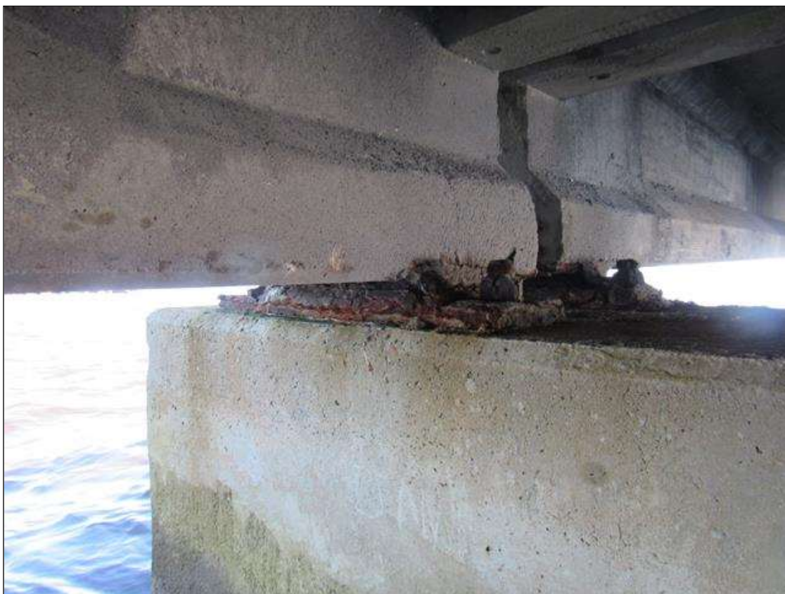
Span 3 Beam 1 Far Bearing: RUST SCALE, BEARING ASSEMBLY.
