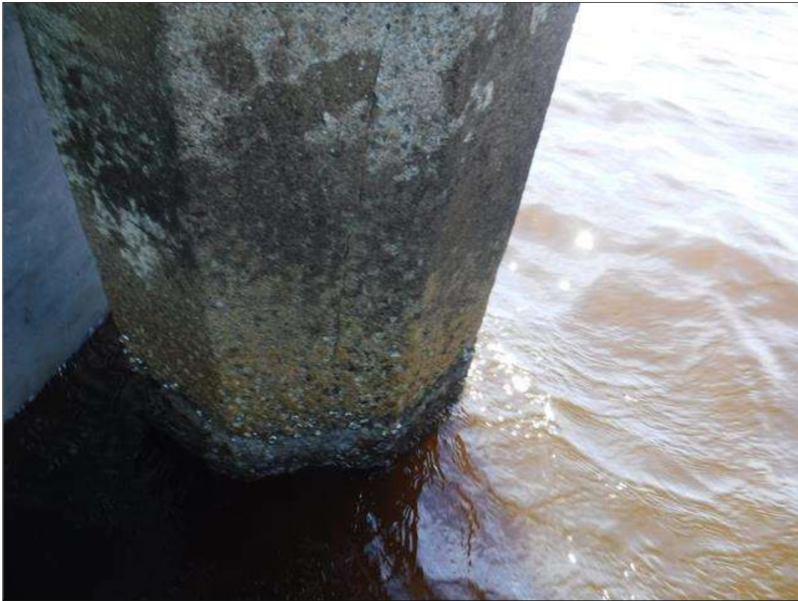
Bent 26 Saved Pile 4: 2' X 1' DELAMINATION, NORTH FACE, 8' FROM BOTTOM OF CAP.
