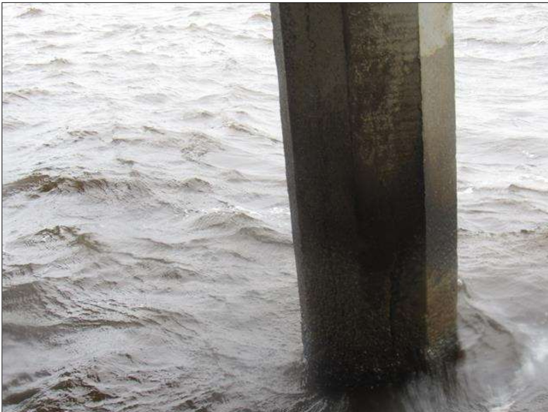
Bent 57 Saved Pile 1: 2' X 1' DELAMINATION, SOUTH FACE, 8' FROM BOTTOM OF CAP.
