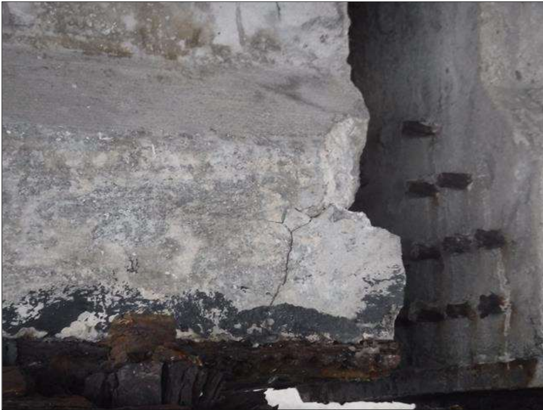
Span 246 Beam 3: (PAR) 6" X 6" X 3" DEEP SPALL WITH EXPOSED STRANDS ON NORTH FACE AT BENT 245
