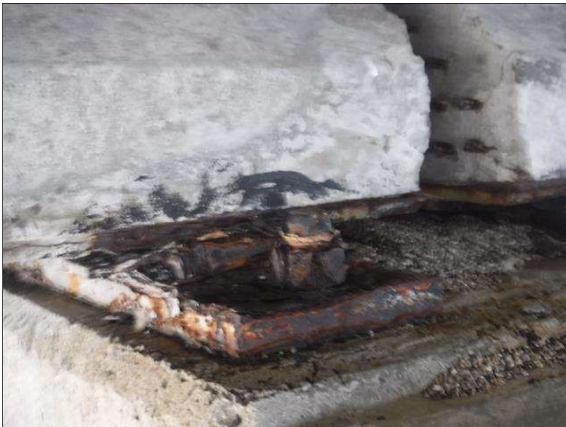
Span 151 Beam 2 Near Bearing: CORROSION WITH LESS THAN 1/16" LOSS. (2" REMAINING).
