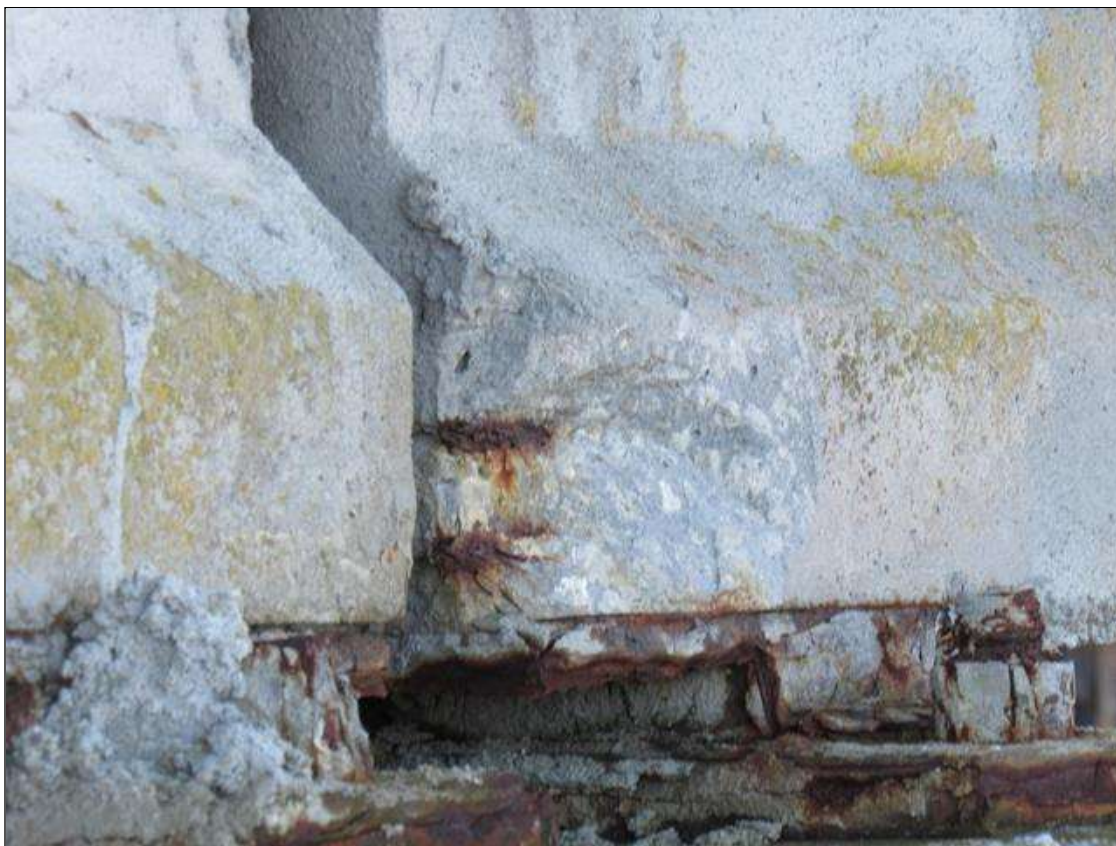
Span 2 Beam 1: (PAR) 8" X 6" X 1" SPALL WITH EXPOSED STRAND, NORTH FACE, AT BENT 2
