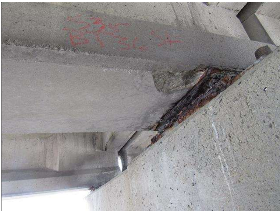
Span 36 Beam 2: 5" DIAMETER X 1" DEEP SPALL ON BOTTOM FACE LOCATED AT BENT 36
