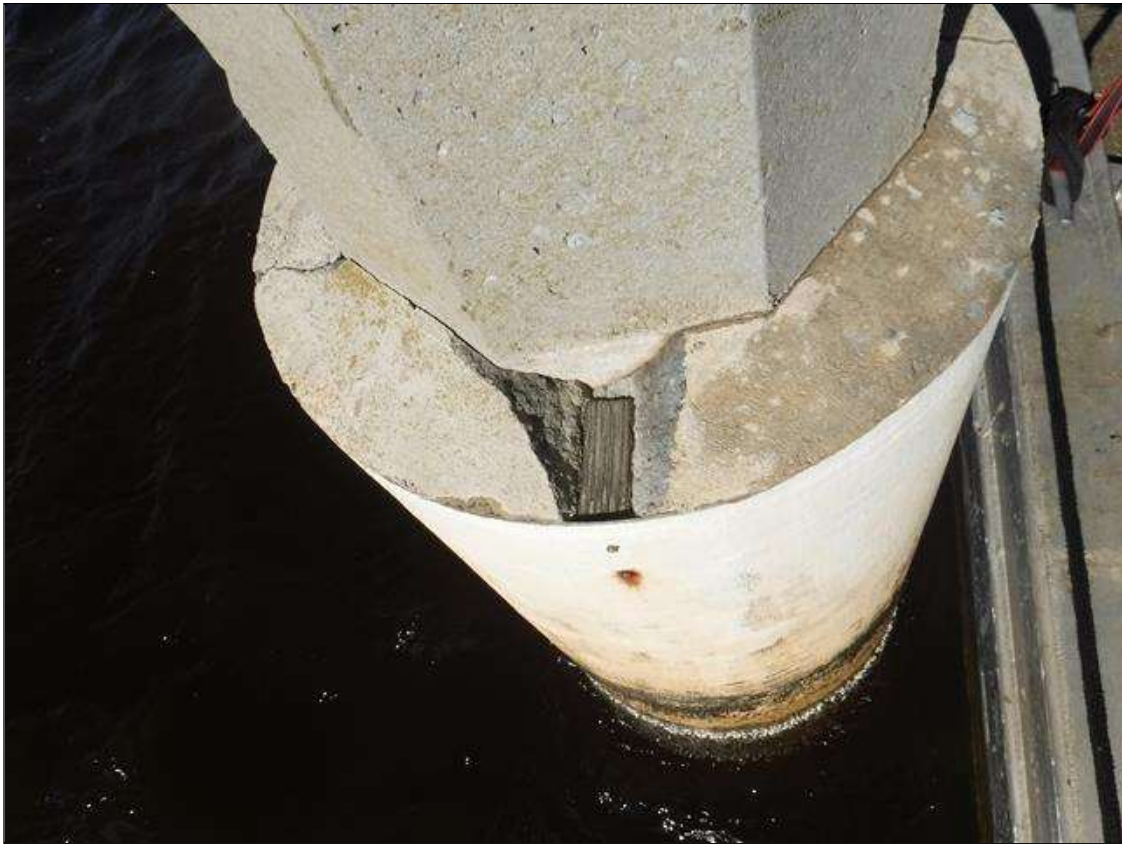
Bent 121 Pile 3: UP TO 6" X 4" X 3" SPALLS, TOP OF PILE JACKET.
