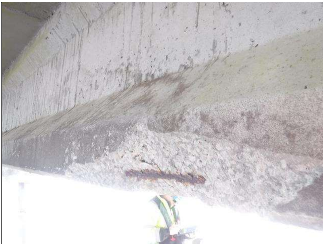
Span 148 Beam 3: (PAR) 3' X 6" X 6" CORNER SPALL, WITH EXPOSED STRAND, BOTTOM FACE, 17' FROM BENT
