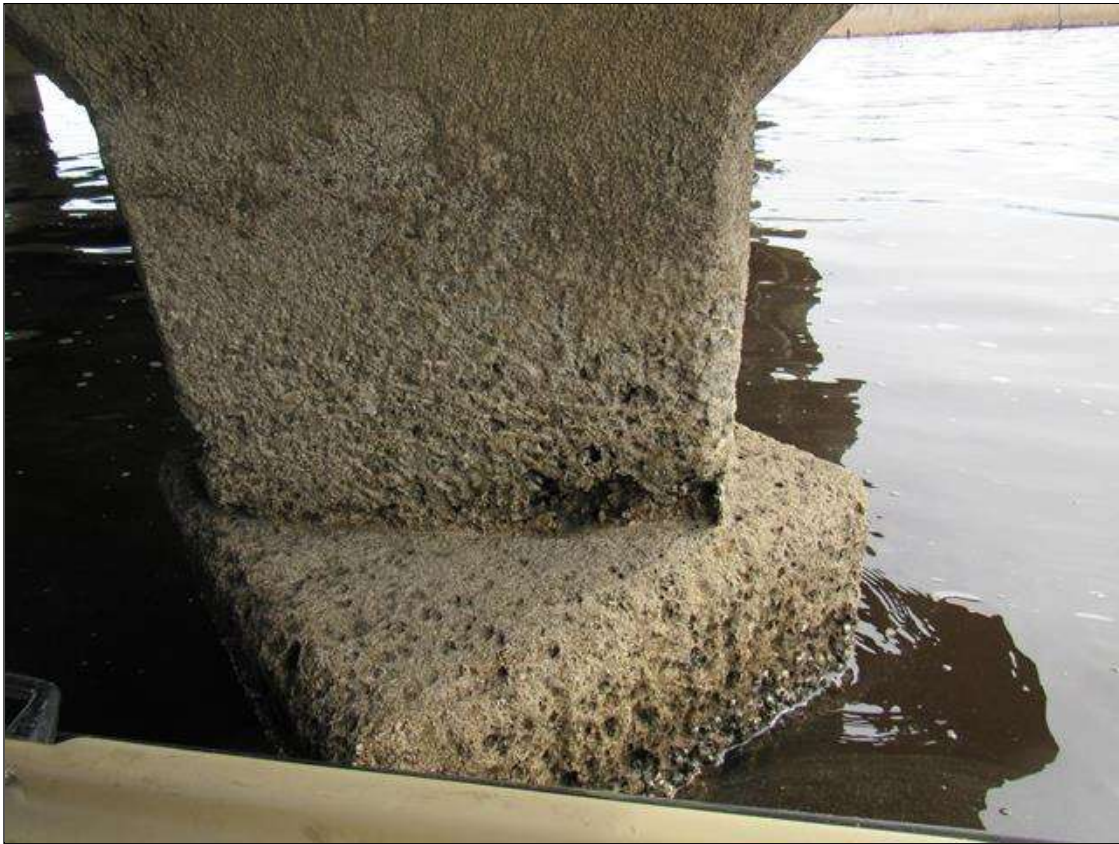
Bent 281 Pile 4: 7" X 3" X 2" DEEP SPALL ON WEST FACE LOCATED AT BOTTOM OF PILE
