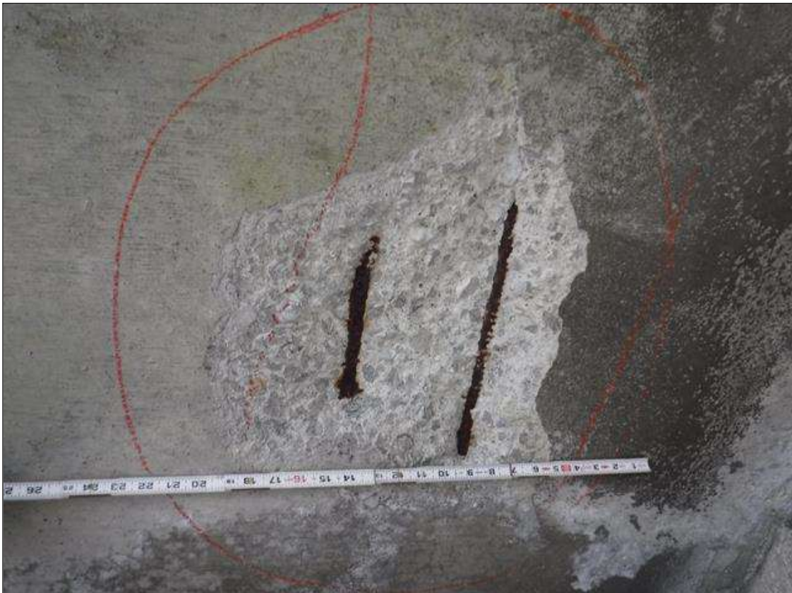
Span 231 Deck: (PAR) 44" DIAMETER X 1 1/2" DEEP SPALL WITH EXPOSED REBAR ON UNDERSIDE OF DECK IN BAY 2 AT BENT 230
