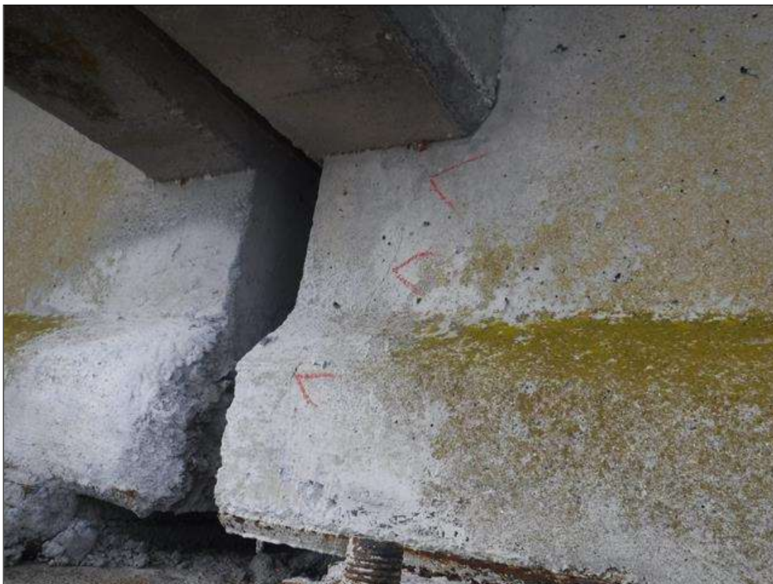
Span 75 Beam 1: 1' HAIRLINE CRACK IN WEB ON NORTH FACE AT BENT 75
