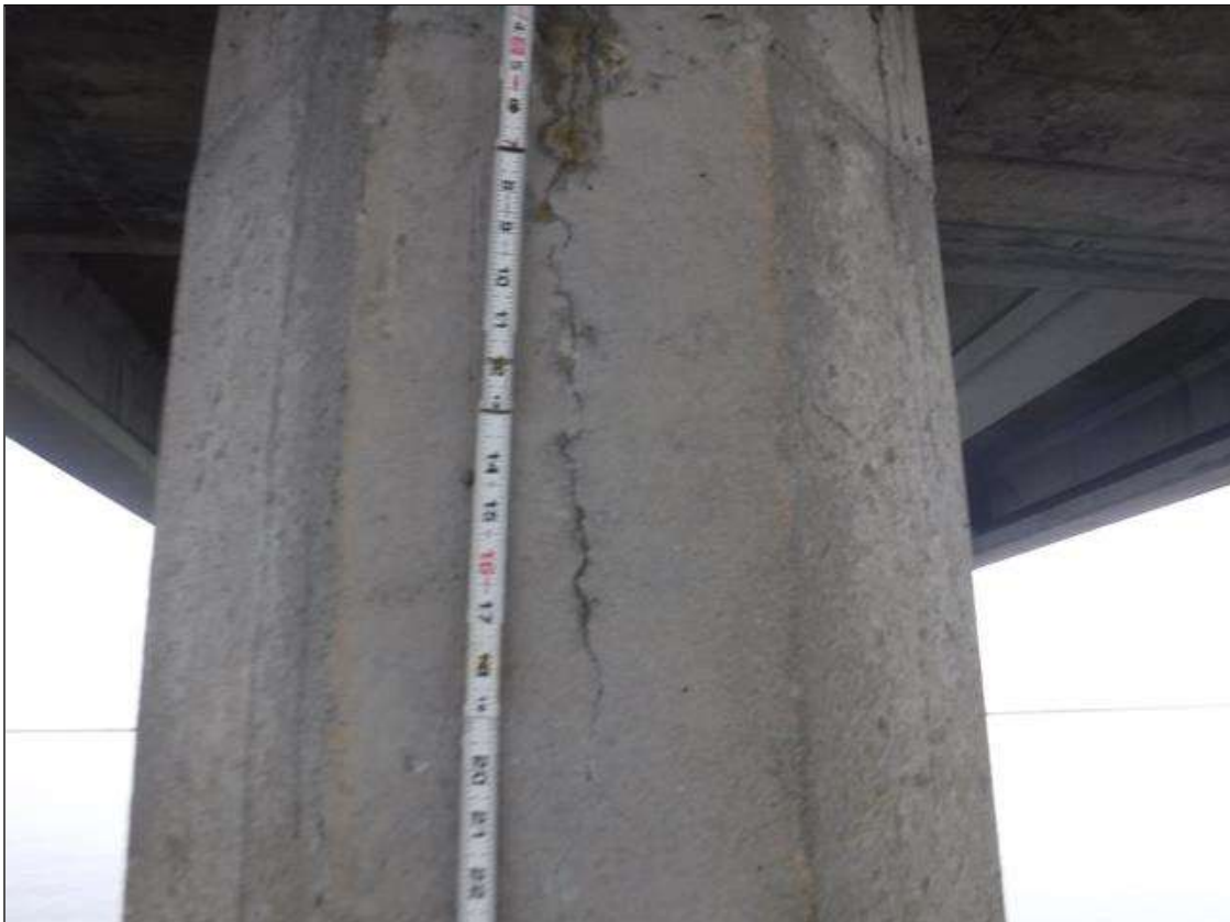
Bent 248 Pile 3: (PAR) HAIRLINE TO 1/16" CRACK FROM BOTTOM OF CAP DOWN 4' ON EAST FACE. SCALING TO 1" DEEP WITH LOOSE AGGREGATE FROM WATERLINE TO MUDLINE.
