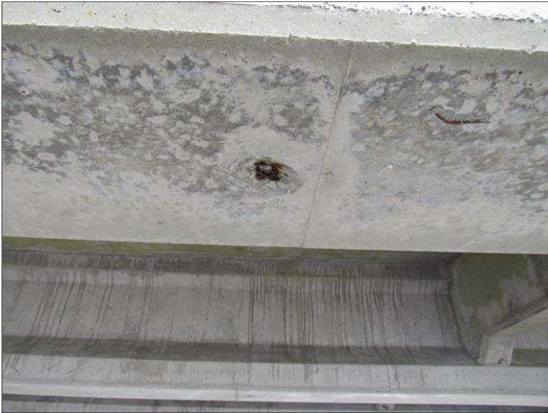
Span 33 Beam 4: 3" DIAMETER X 1/2" DEEP SPALL ON BOTTOM FACE AT MIDSPAN
