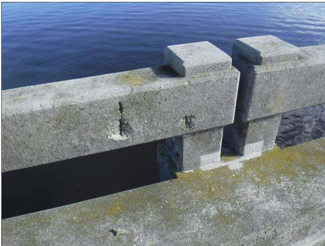
Span 264 Left Bridge Rail: (2) UP 4" X 8" X 3/4" SPALLS WITH EXPOSED REBAR ON RIGHT FACE LOCATED 1' BEFORE POST 3
