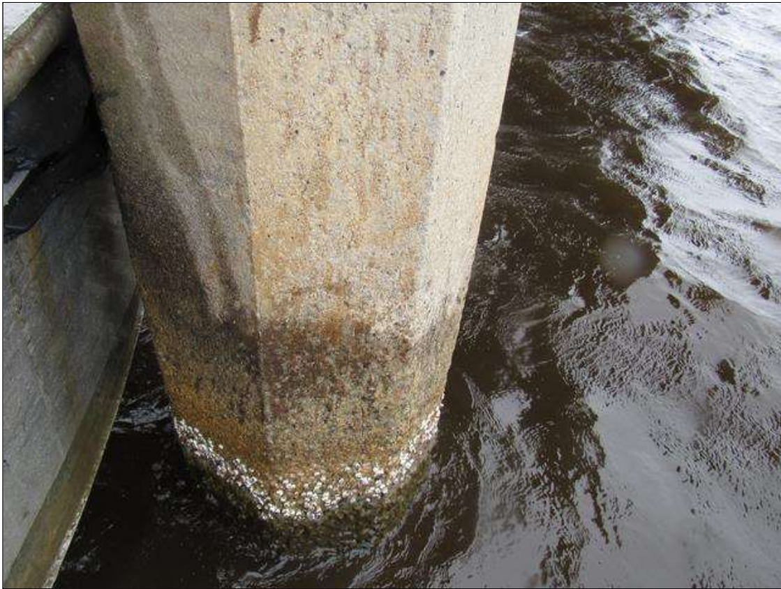
Bent 77 Pile 6: (PAR) UP TO 1' X 0.06" VERTICAL CRACK, SOUTH FACE, BEGINNING 9' FROM BOTTOM OF CAP.
