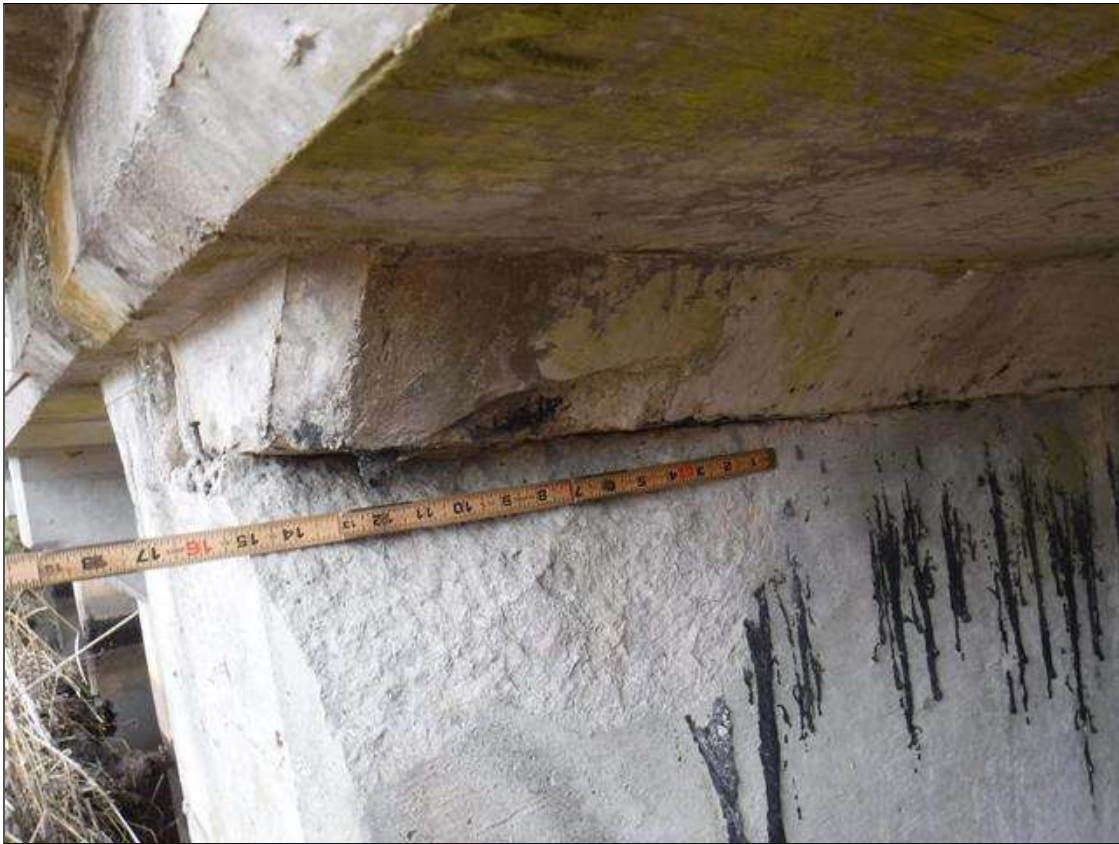
Bent 331 Cap 1: 15" X 7" X 4" SPALL, EAST FACE, SOUTH END OF CAP.
