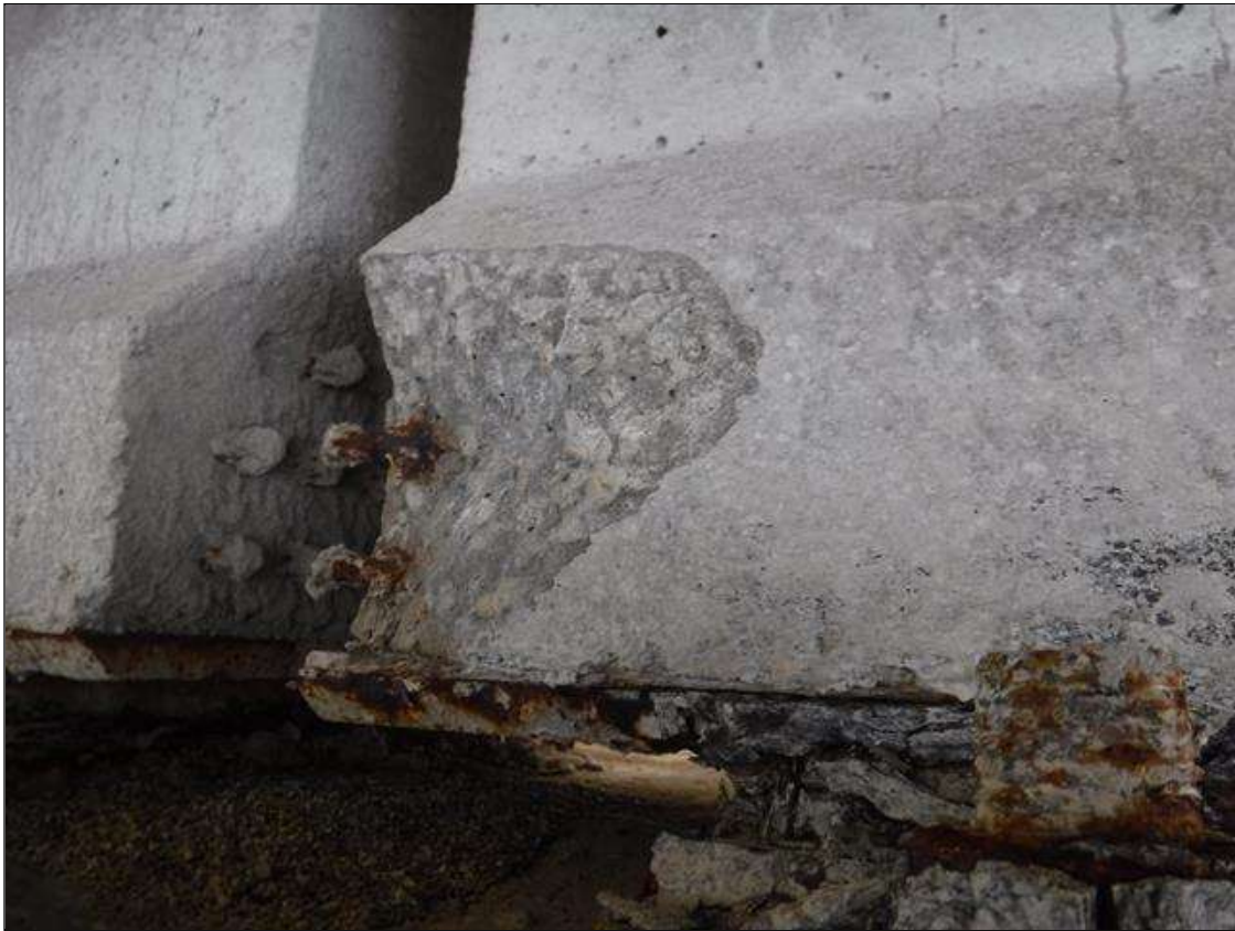
Span 224 Beam 3: (PAR) 6" X 6" X 3" DEEP SPALL WITH EXPOSED STRAND ON BOTTOM FLANGE NORTH FACE AT BENT 224
