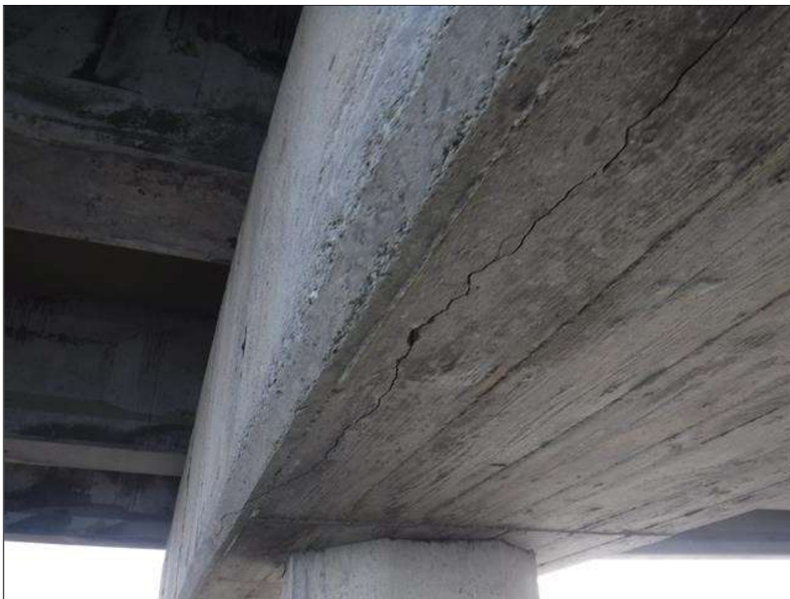
Bent 128 Cap 1: 6' X 1/16" CRACK ON EAST BOTTOM FACE BETWEEN PILES 1 AND 2
