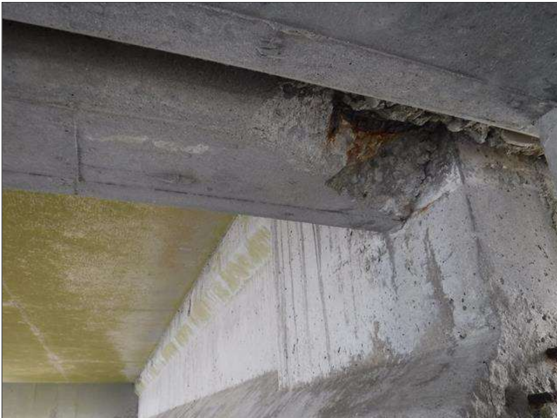
Span 107 Beam 3: (PAR) 1' X 6" X 4" DEEP SPALL WITH EXPOSED REBAR AND 10 PERCENT SECTION LOSS IN BAY 3 DIAPHRAGM AT BENT 106
