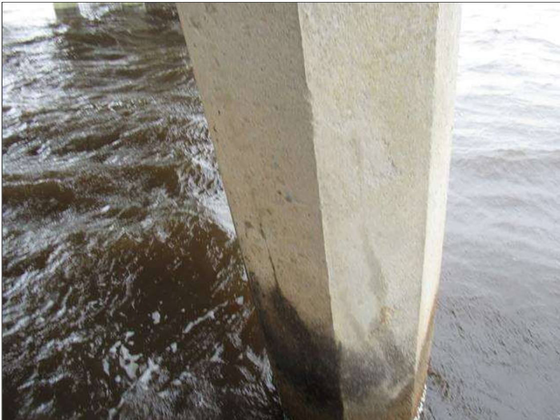
Bent 101 Pile 6: (PAR) 3' X 1/8" CRACKS ON NORTH FACE WITH SURROUNDING DELAMINATION 3' X 1', 10' FROM BOTTOM OF CAP
