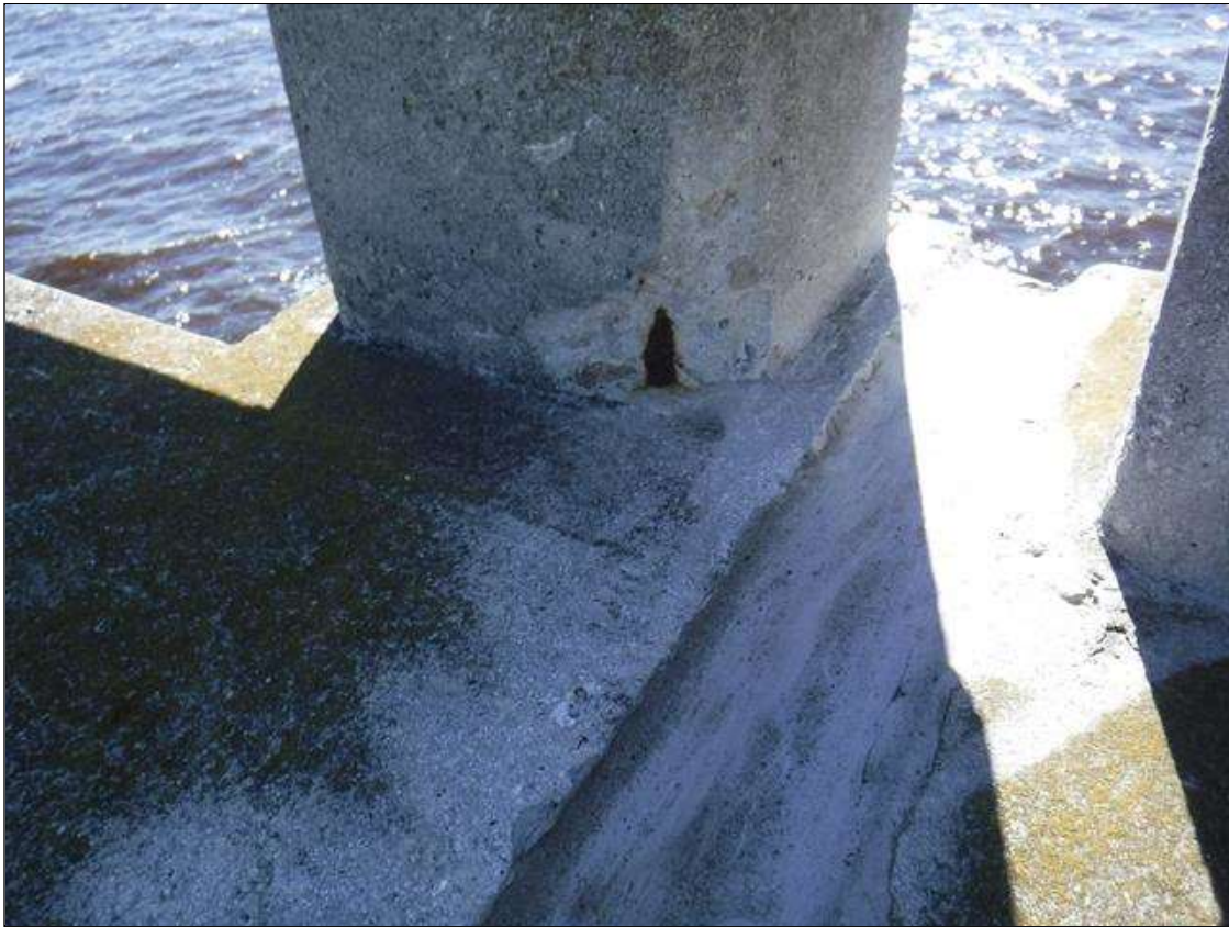
Span 82 Right Bridge Rail: 4" X 2 1/2" X 5" SPALL WITH EXPOSED REBAR AT BOTTOM LEFT CORNER LOCATED AT POST 1
