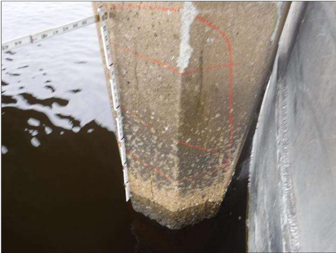
Bent 249 Pile 3: (PAR) (3) UP TO 4' X 0.25" VERTICAL CRACKS WITH 4' X 2' SURROUNDING DELAMINATION ON NORTH FACE, BEGINNING 6' BOTTOM OF CAP
