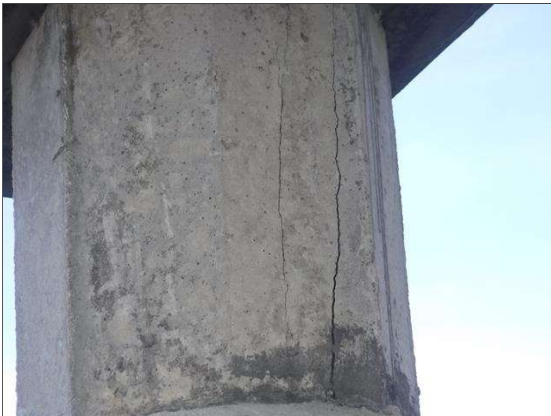
Bent 131 Pile 1: (PAR) 1' X UP TO 0.16" VERTICAL CRACKS, AT RANDOM THROUGHOUT.
