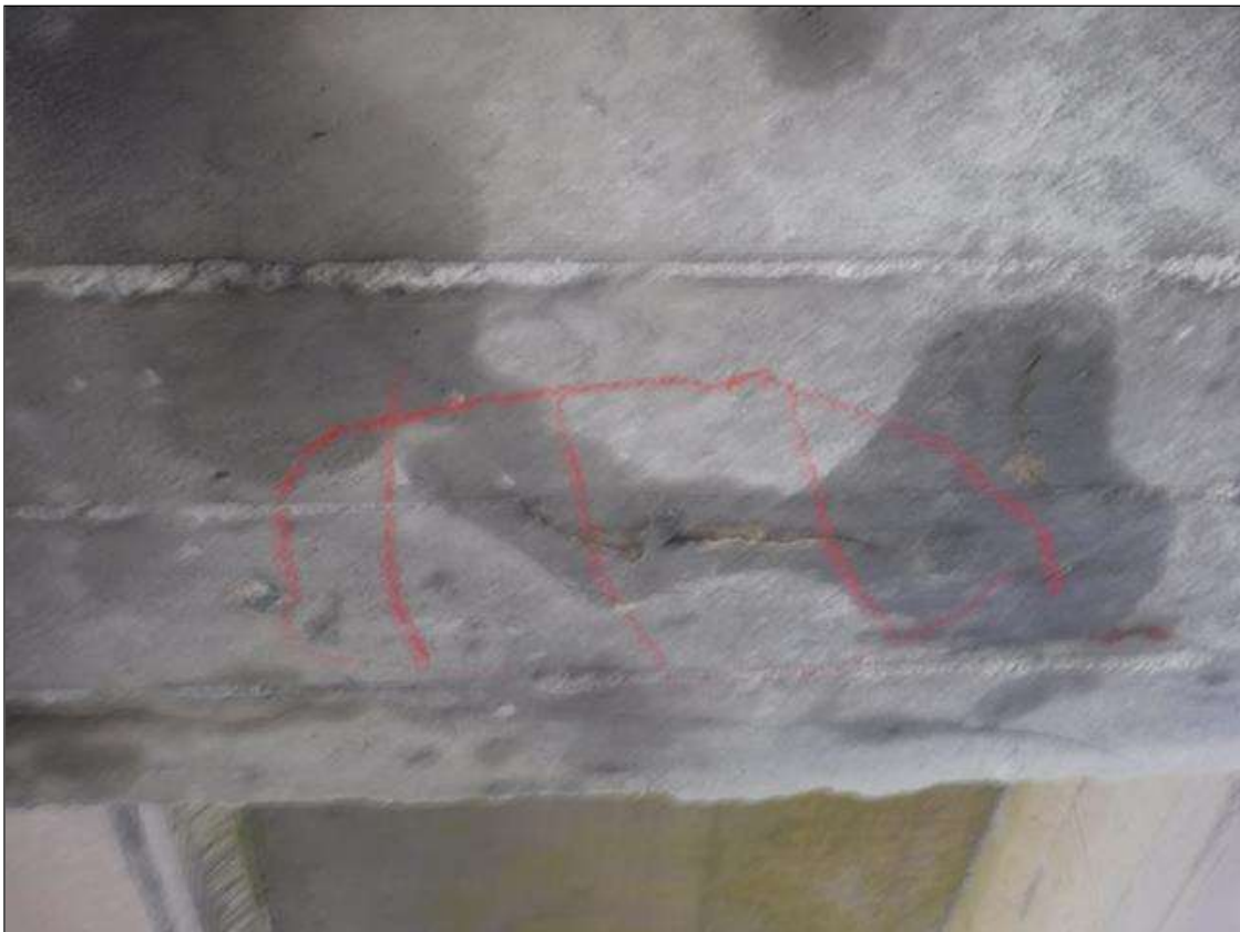
Bent 164 Cap 1: 7' X UP TO 1/32" LONGITUDINAL CRACK WITH 1' DIAMETER DELAMINATION ON BOTTOM OF CAP, BETWEEN BEAMS 1 AND 2.
