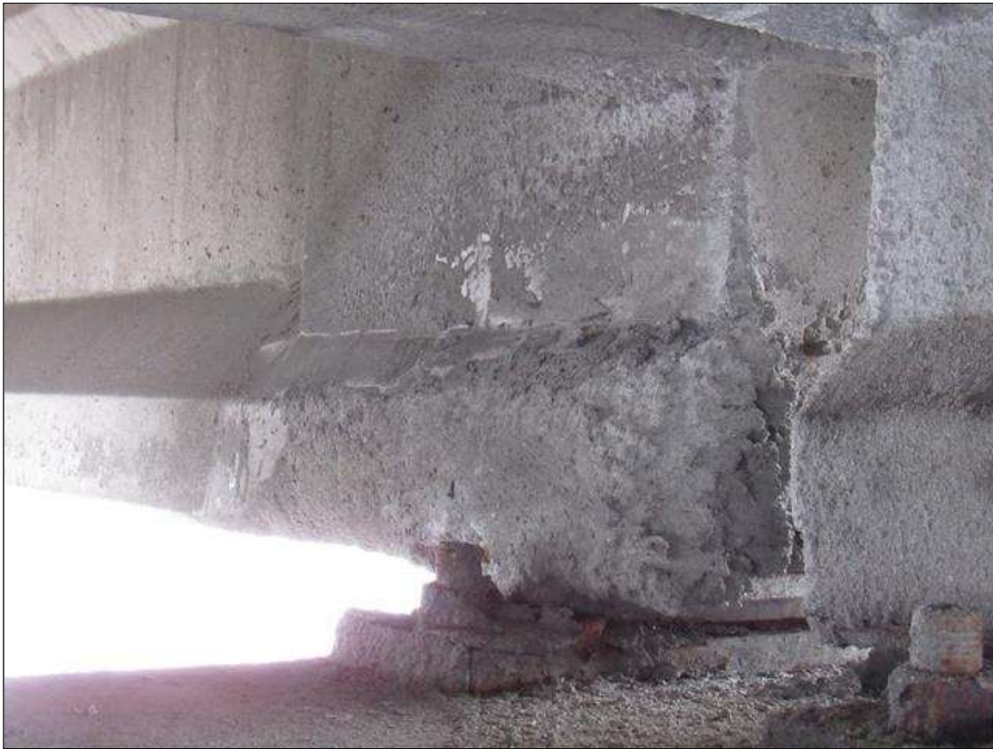
Span 38 Beam 4: 2.5' X UP TO 8" PATCHED AREA, BOTTOM FACE, EXTENDING 10" ONTO NORTH FACE, AT BENT 37.
