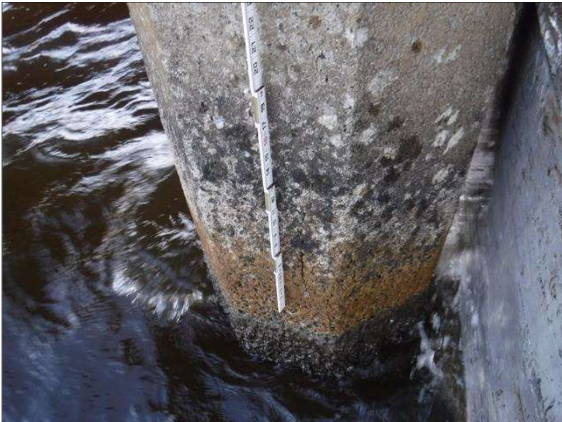
Bent 120 Saved Pile 2: 3' X 1' DELAMINATION, NORTH FACE, 9' FROM BOTTOM OF CAP, EXTENDING BELOW WATERLINE.
