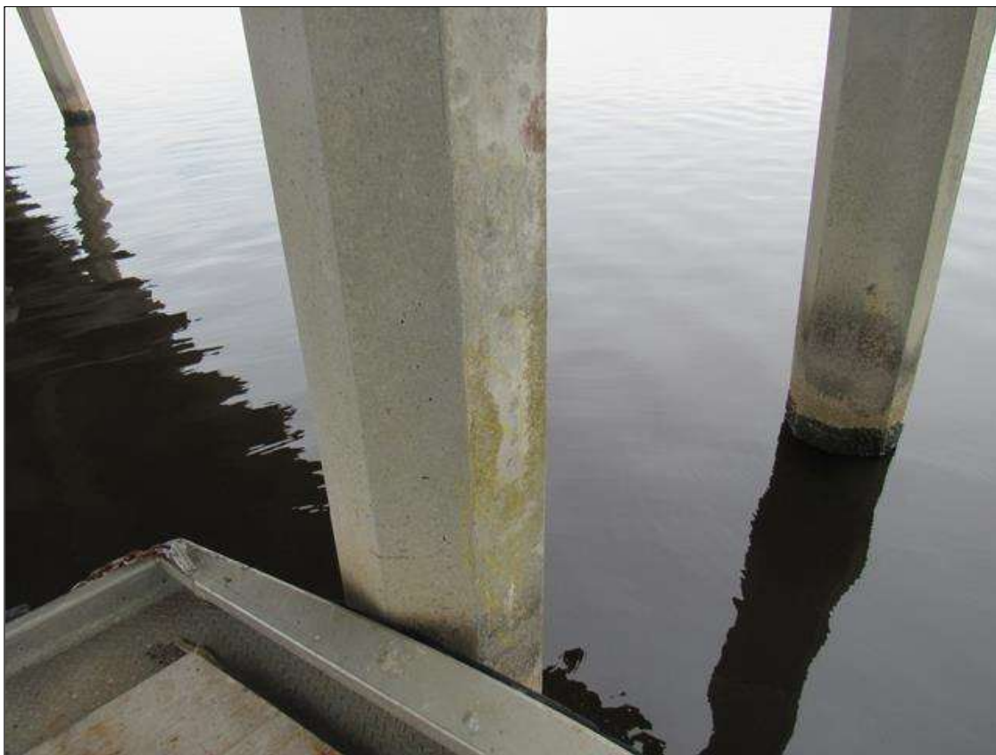
Bent 31 Saved Pile 3: 4' X UP TO 1' DELAMINATION, WEST FACE, 5' FROM BOTTOM OF CAP.
