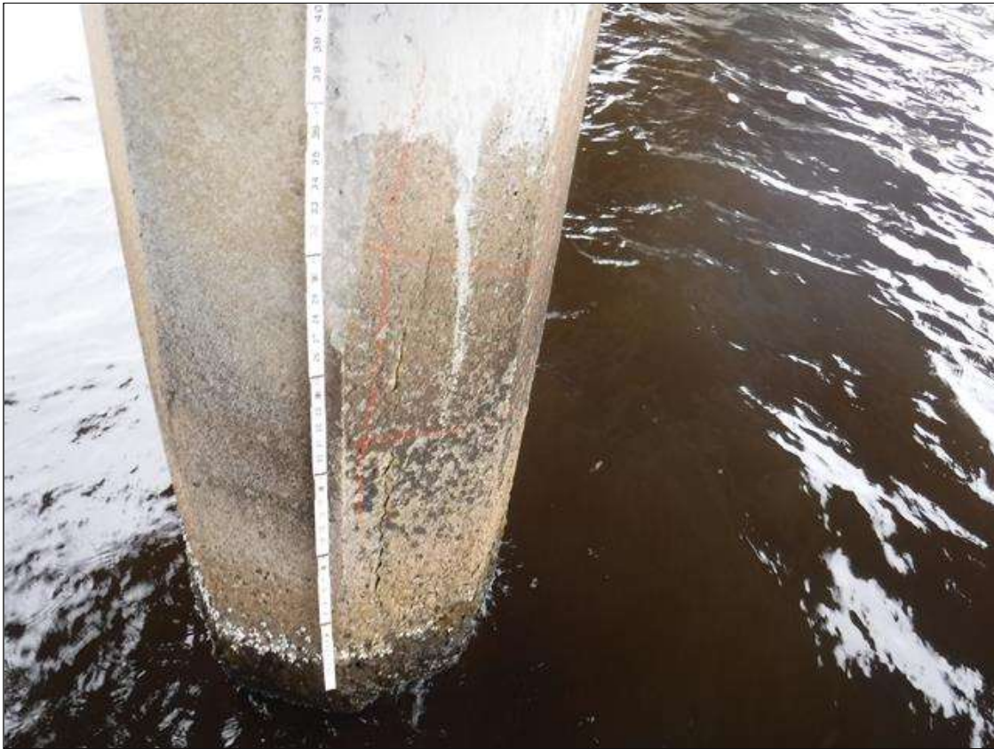
Bent 252 Pile 3: (PAR) (2) UP TO 2' X 0.0125" VERTICAL CRACKS, NORTH FACE, 8' FROM BOTTOM OF CAP, WITH ADJACENT 2' X 3' DELAMINATION.
