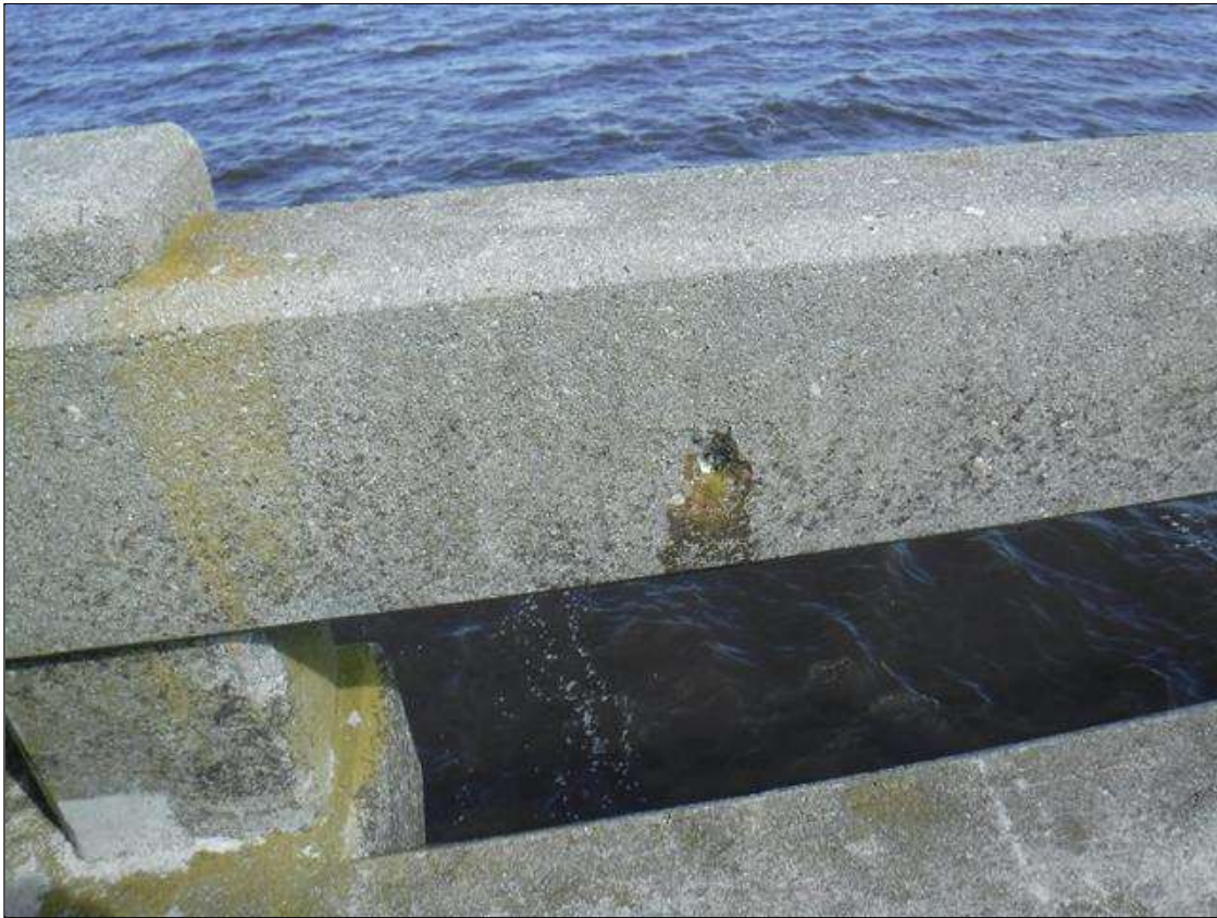
Span 180 Left Bridge Rail: 4" X 6" FAILED PATCHED AREA, SOUTH FACE, BETWEEN RAIL POSTS 7 AND 8 FROM BENT 179.
