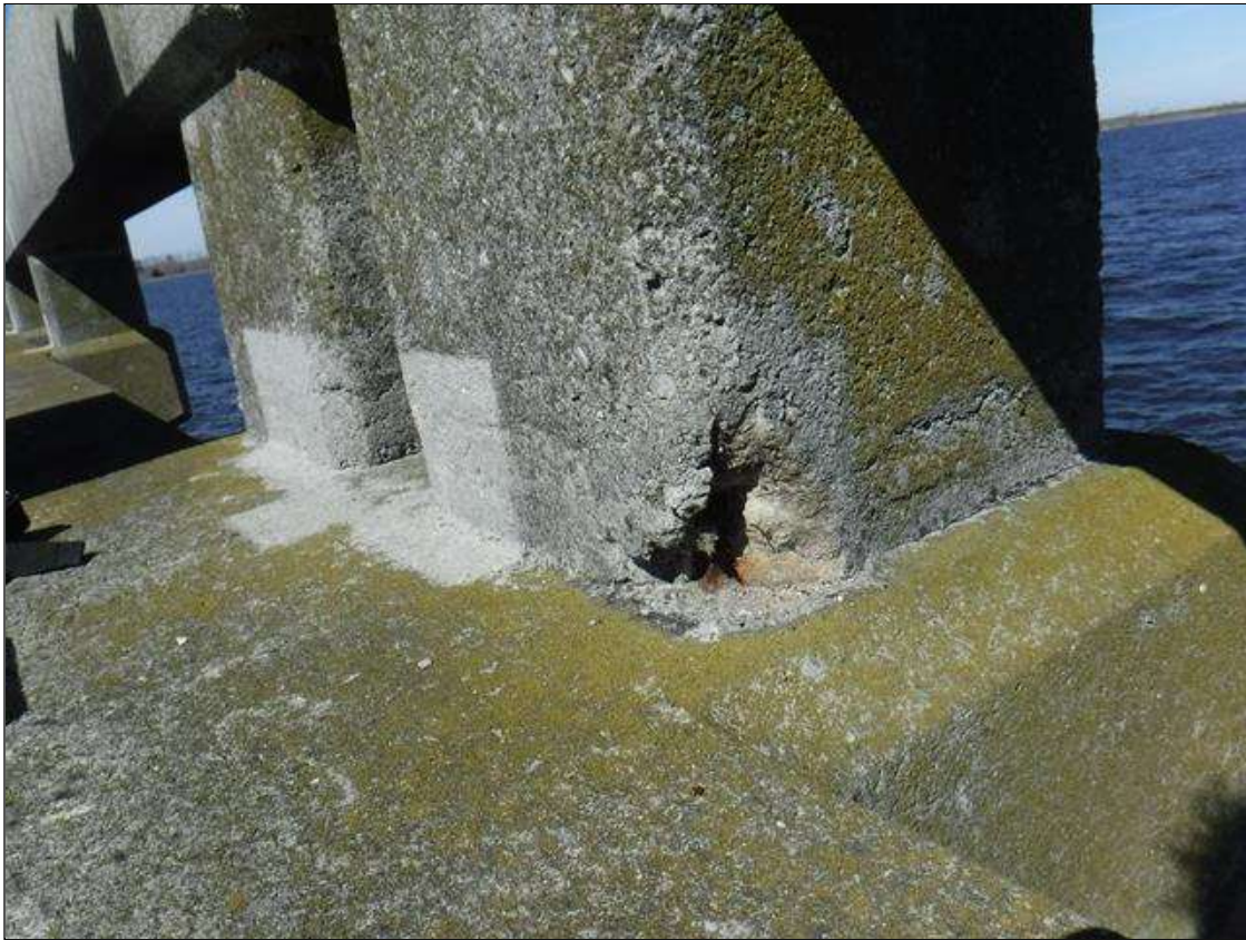
Span 66 Left Bridge Rail: 3" X 3" X 2" SPALL WITH EXPOSED REBAR AT BOTTOM RIGHT CORNER LOCATED AT POST 4
