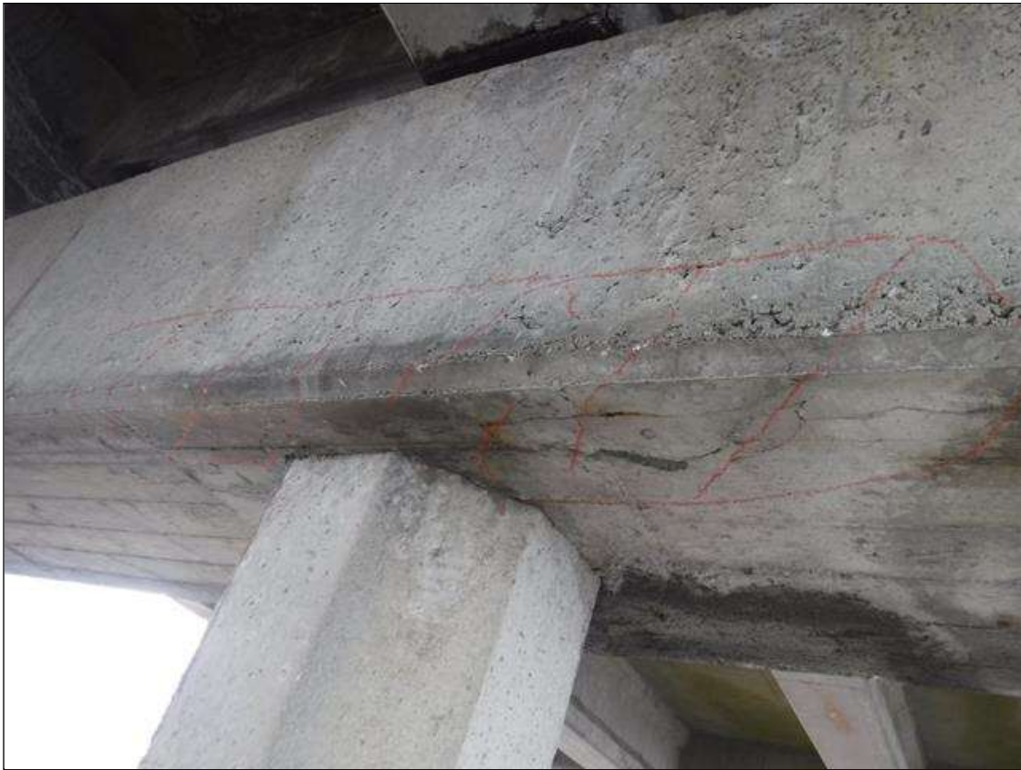
Bent 188 Cap 1: 6' X 8" X 12" DEEP DELAMINATION ON BOTTOM AND EAST FACE AT PILE
