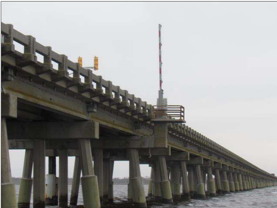
TRAFFIC GATE ON NORTH OVERHANG OF BENT 110
