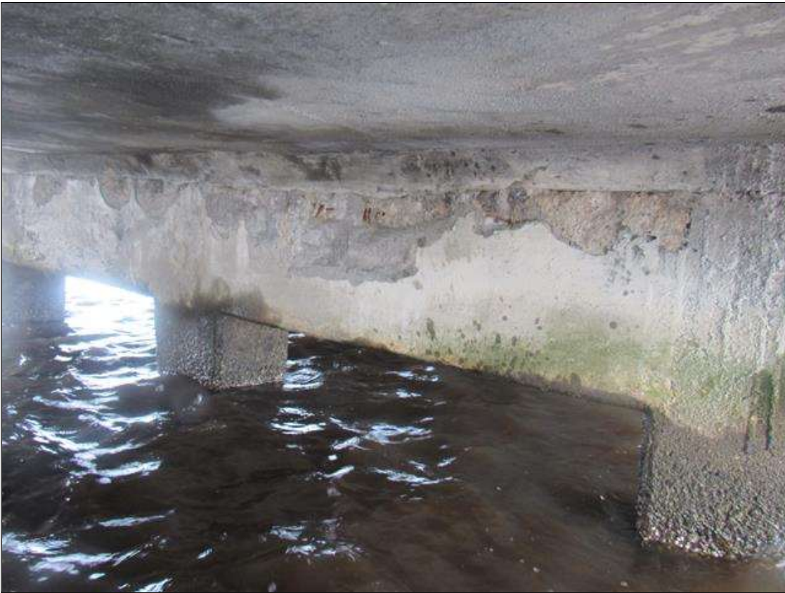
Bent 295 Cap 1: (PAR) 12' X UP TO 14" HIGH X 5" DEEP SPALL WITH EXPOSED REBAR ON EAST FACE LOCATED BETWEEN PILES 1 AND 3. LOSS OF UP TO 5" OF BEARING AREA FOR SLAB
