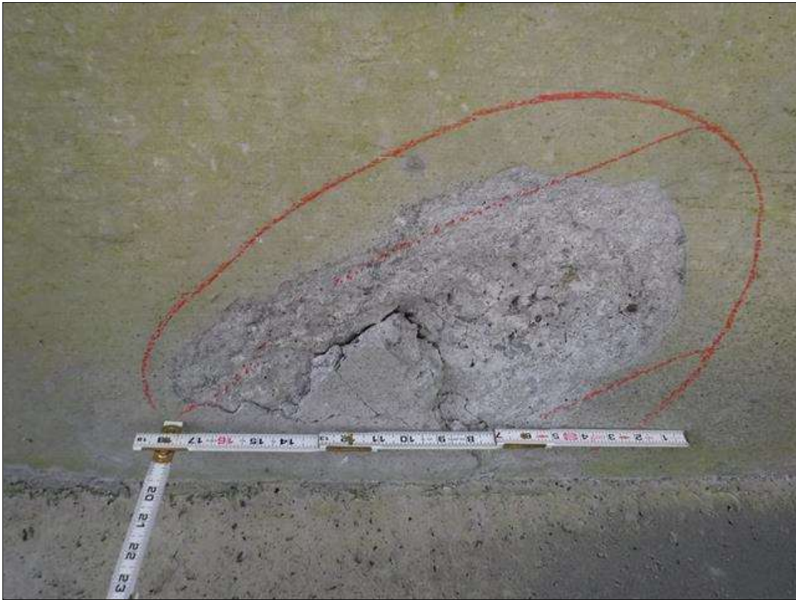
Span 208 Deck: 16" DIAMETER X 2" DEEP SPALL IN UNDERSIDE OF DECK, 5' FROM BENT 207, ADJACENT TO BEAM 4
