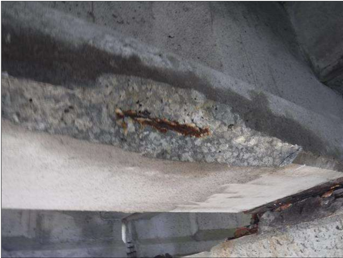
Span 166 Beam 3: (PAR) 2' X 6" X 2" DEEP SPALL WITH EXPOSED STRAND ON BOTTOM FLANGE 2' FROM BENT 165. STRAND HAS 10% SECTION LOSS
