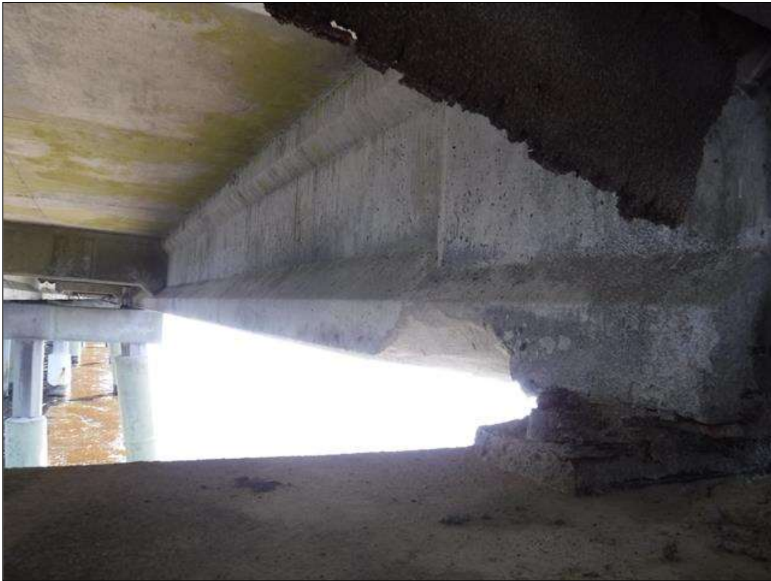
Span 142 Beam 4: 36" X 8" PATCHED AREA, NORTH FACE, AT BENT 141.
