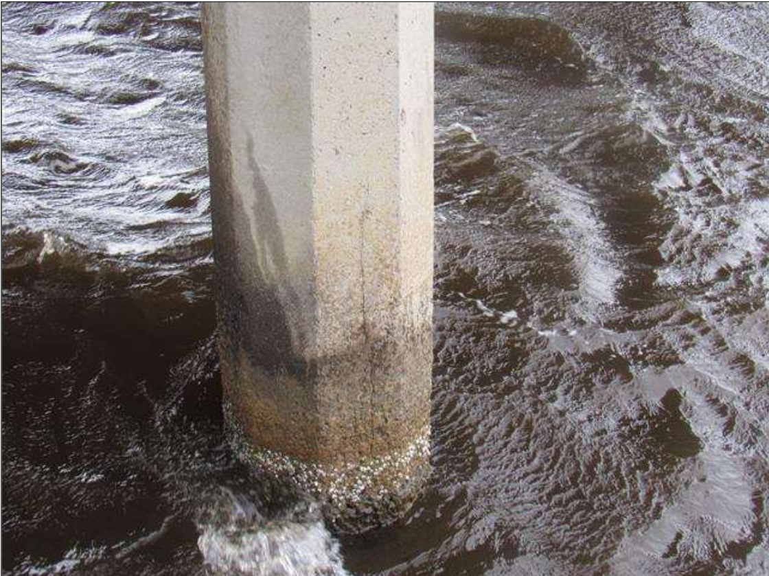
Bent 82 Pile 4: (PAR) (3) UP TO 3' X 1/16" VERTICAL CRACKS, BEGINNING 8' FROM BOTTOM OF CAP, AT RANDOM THROUGHOUT.
