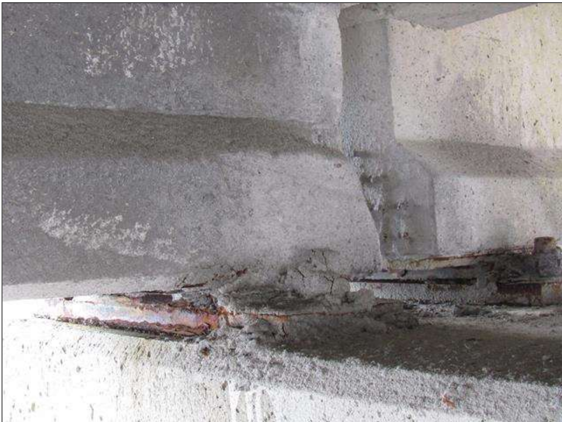
Span 59 Beam 1: 7" X 10" PATCHED AREA, SOUTH FACE, AT BENT 59.
