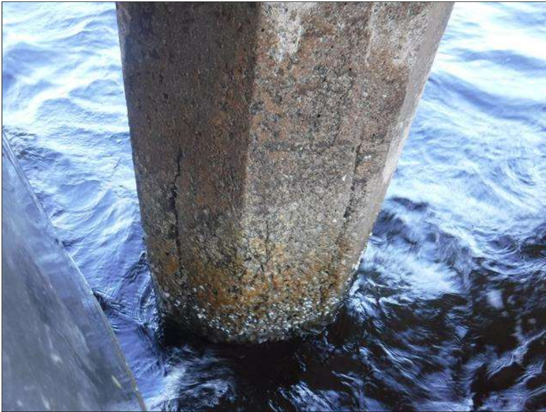
Bent 25 Saved Pile 2: 2' X 8" DELAMINATION, SOUTH FACE, BEGINNING 8' FROM BOTTOM OF CAP AND EXTENDING BELOW WATERLINE.
