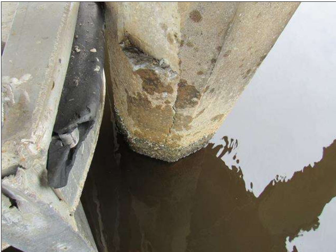
Bent 33 Saved Pile 2: (PAR) HAIRLINE TO 1/16" CRACK WITH ADJACENT DELAMINATION, 8' BELOW CAP, DOWN 6', SOUTH FACE. SCALING TO 1" DEEP WITH LOOSE AGGREGATE FROM WATERLINE TO MUDLINE.
