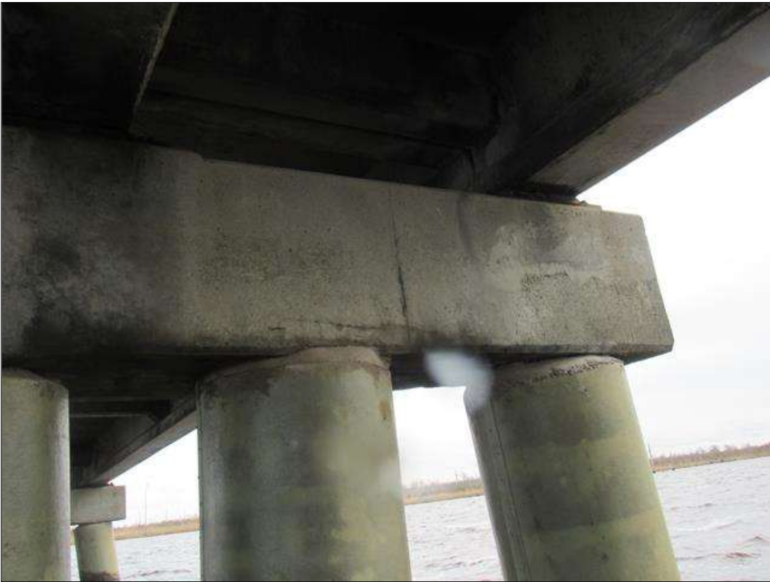
Bent 269 Cap 1: 3' LONG HORIZONTAL CRACK UP TO 1/16" WIDE ON NEAR FACE LOCATED ABOVE PILE 5
