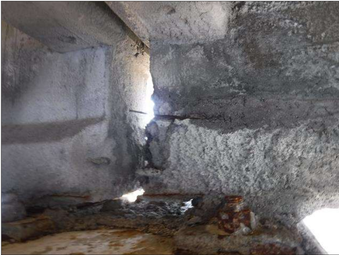
Span 23 Beam 4: 30" X 12" PATCHED AREA ON NORTH FACE, AT BENT 23.
