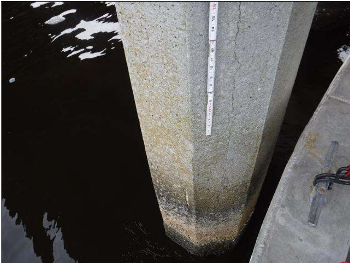
Bent 229 Pile 1: (PAR) (4) UP TO 6' X 0.014' VERTICAL CRACKS, NORTH FACE, 7' FROM BOTTOM OF CAP, WITH ADJACENT 2' X 1' DELAMINATION.
