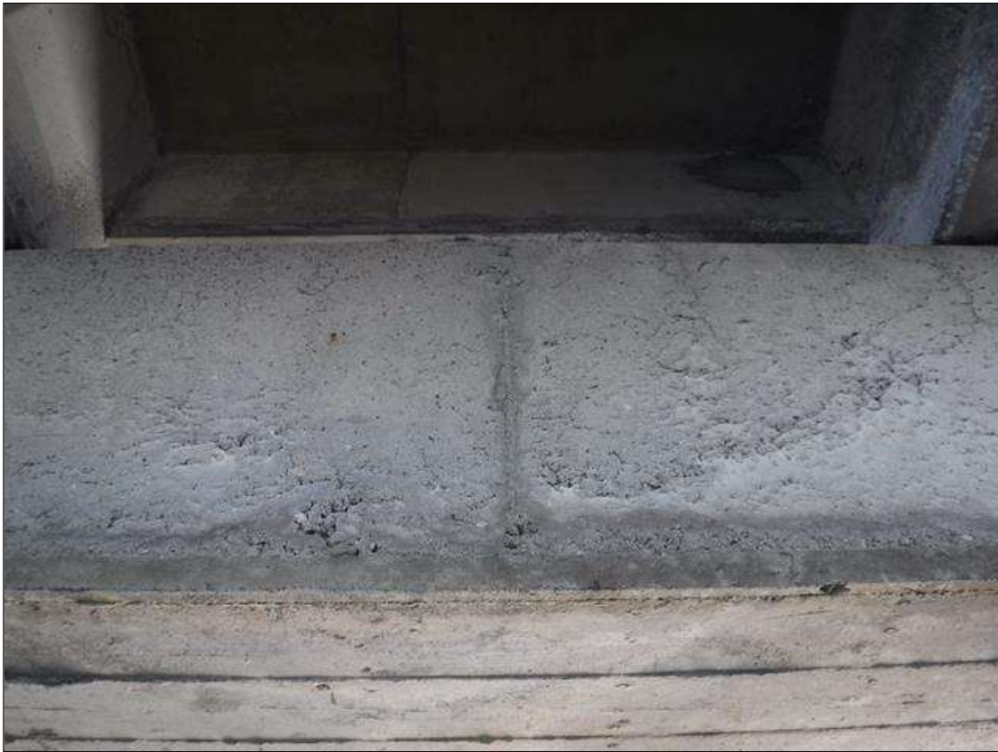
Bent 154 Cap 1: 7' X 3' AREA OF HONEYCOMBING, WEST FACE, BETWEEN BEAMS 2 AND 3.
