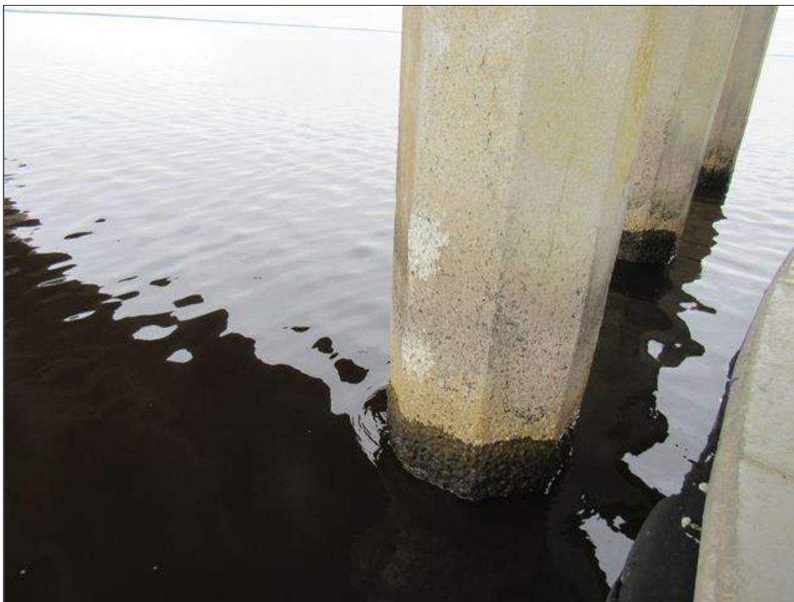
Bent 36 Saved Pile 2: (2) UP TO 4" X 4" X 1" SPALLS, NORTH FACE, 8' FROM BOTTOM OF CAP.
