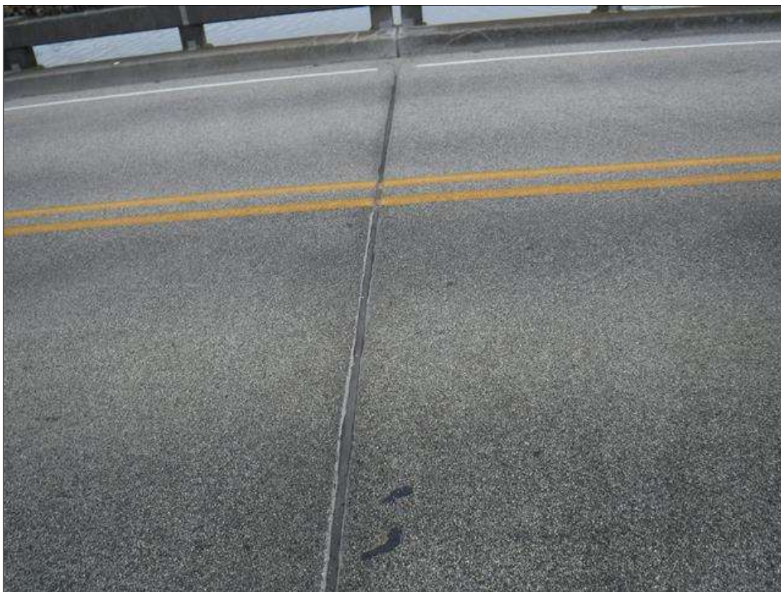
TYPICAL JOINT, BENT 2 JOINT SHOWN
