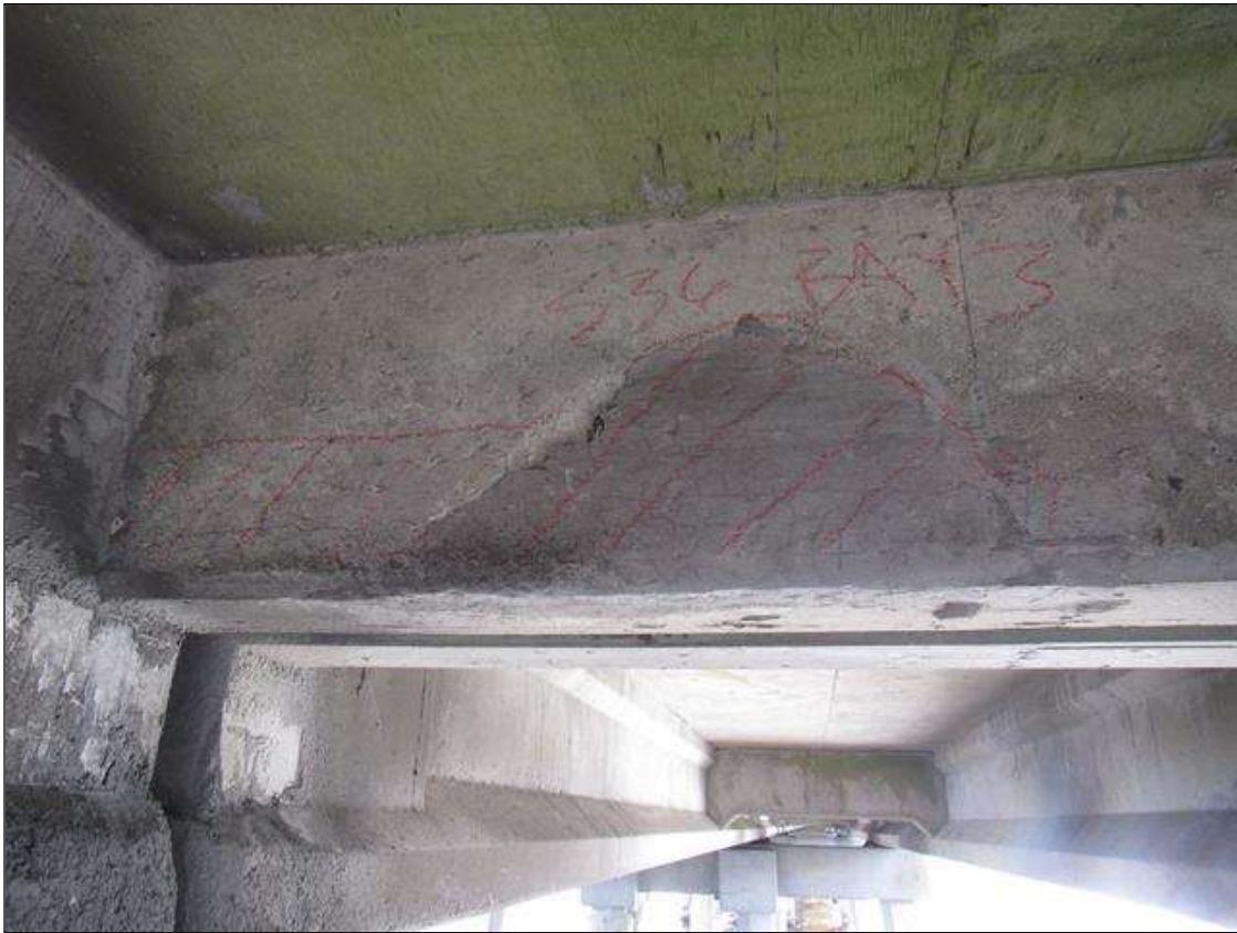
Span 36 Beam 3: 3' X UP TO 10" X 1' CRACKED PATCHED AREA, WEST FACE, END DIAPHRAGM, BETWEEN BEAMS 3 AND 4, AT BENT 36.
