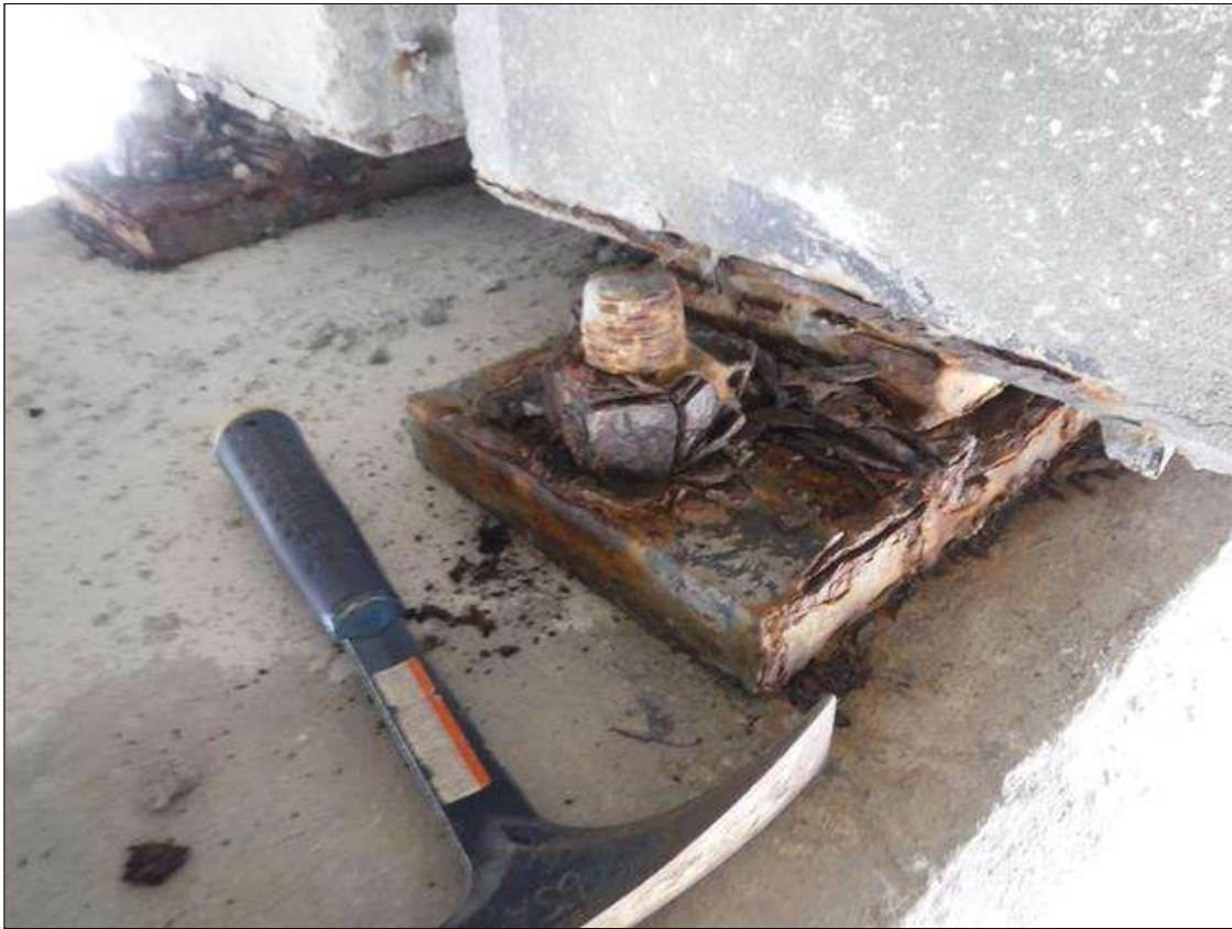
Span 231 Beam 2 Near Bearing: CORROSION WITH LESS THAN 1/16" LOSS. (2" REMAINING).
