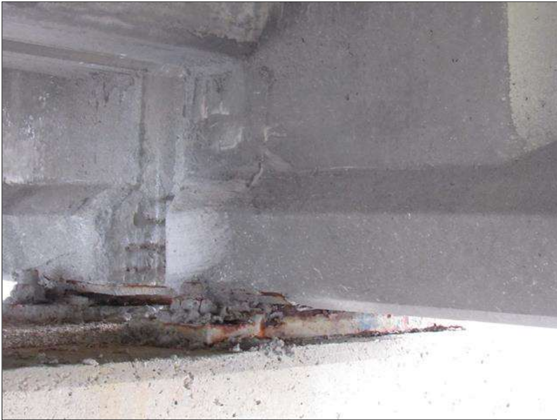
Span 53 Beam 4: 12" X 12" PATCHED AREA, NORTH FACE, AT BENT 53.
