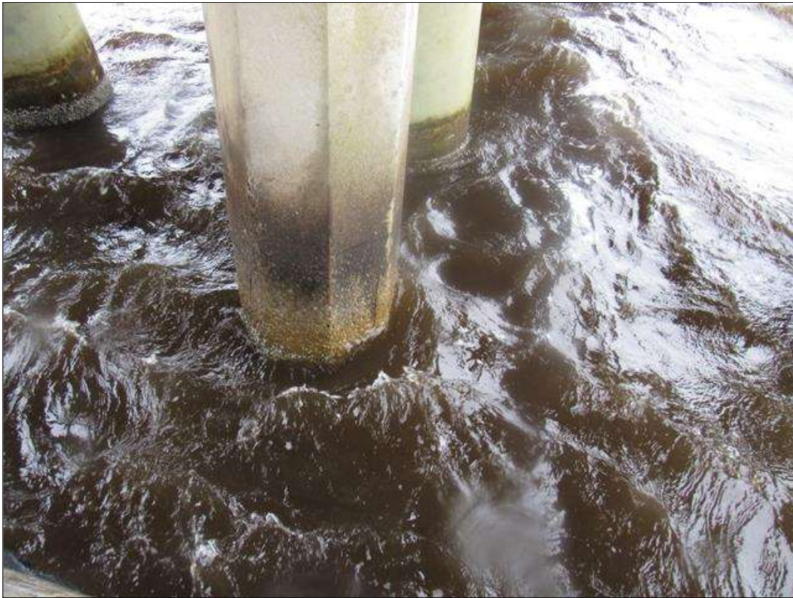
Bent 73 Pile 3: (PAR) (3) UP TO 2' X 0.25" VERTICAL CRACKS WITH RUST STAINING AND SURROUNDING DELAMINATION, BEGINNING 8' FROM BOTTOM OF CAP, AT RANDOM THROUGHOUT.
