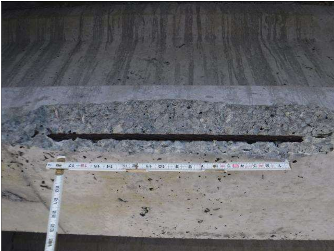
Span 209 Beam 2: (PAR) 32" X 3 X 3" CORNER SPALL, WITH EXPOSED STRAND, BOTTOM NORTH CORNER, 20' FROM BENT 208.
