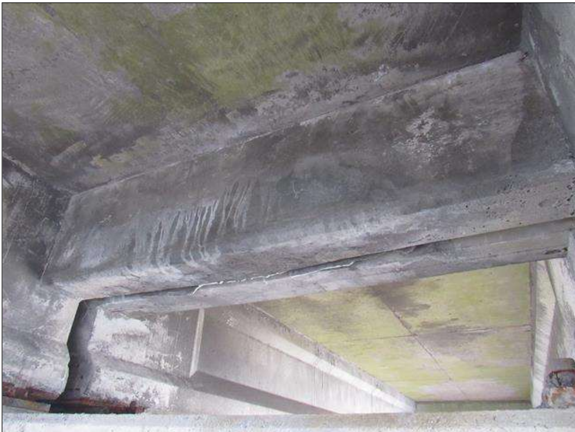
Span 34 Beam 3: 7' X UP TO 9" X 1' PATCHED AREA, END DIAPHRAGM, BETWEEN BEAMS 3 AND 4, AT BENT 34.
