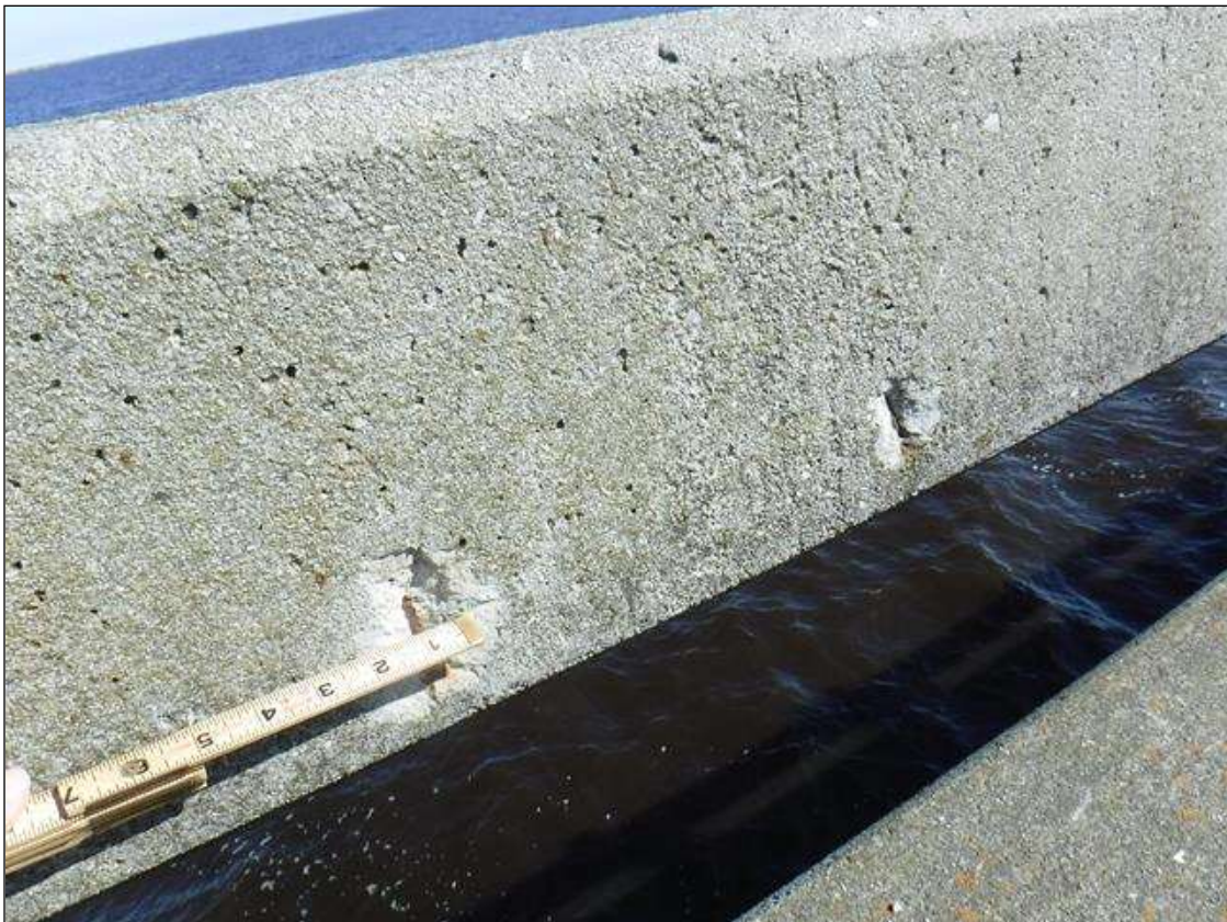
Span 37 Left Bridge Rail: (2) 3" DIAMETER SPALLS WITH EXPOSED REBAR ON RIGHT FACE LOCATED AT MIDSPAN
