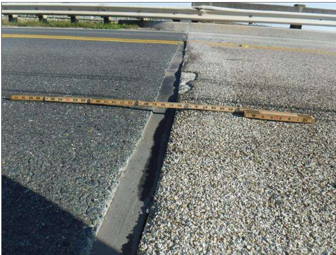
1/2" SETTLEMENT IN JOINT BETWEEN NEAR APPROACH AND SPAN 1, 3' FROM RIGHT LANE
