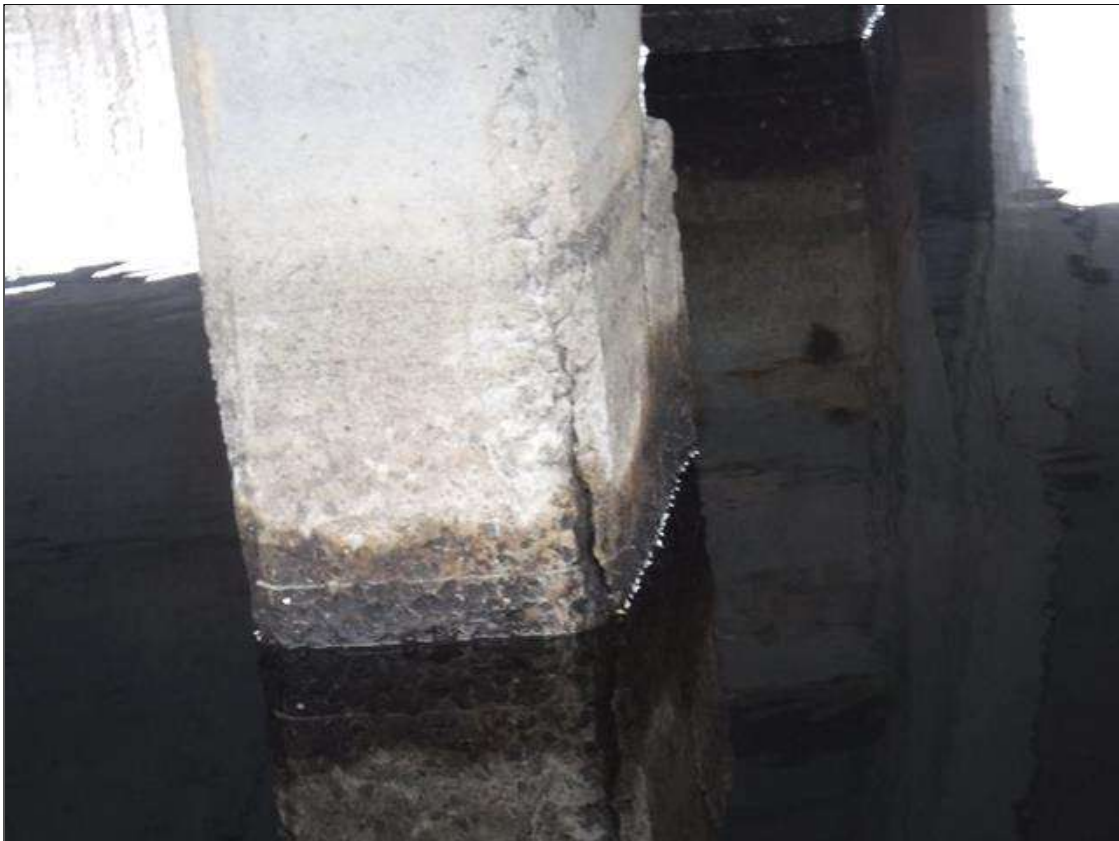
Bent 336 Pile 3: 18" X 4" X 1" SPALL, WITH EXPOSED REINFORCING, NORTHEAST CORNER.
