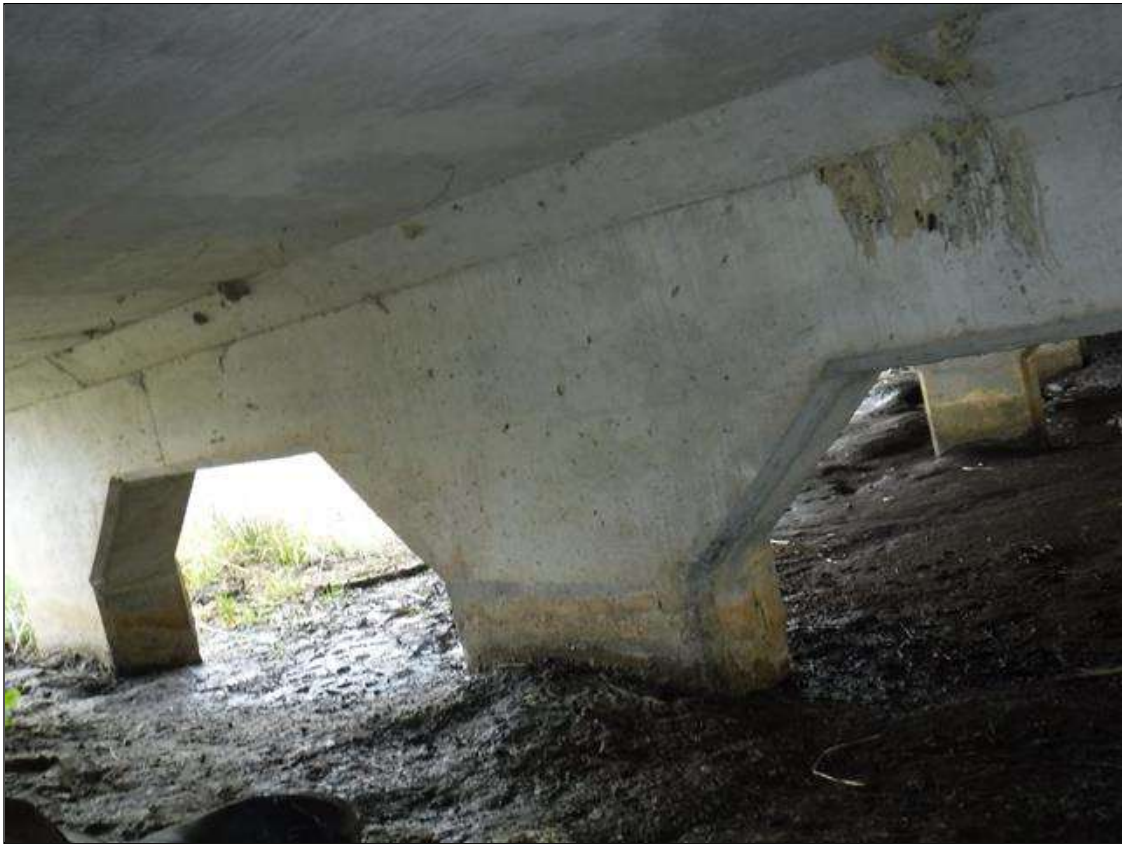
Bent 342 Cap 1: 4' LONG X UP TO 1/16" WIDE LONGITUDINAL CRACK ON EAST FACE LOCATED ABOVE PILE 3
