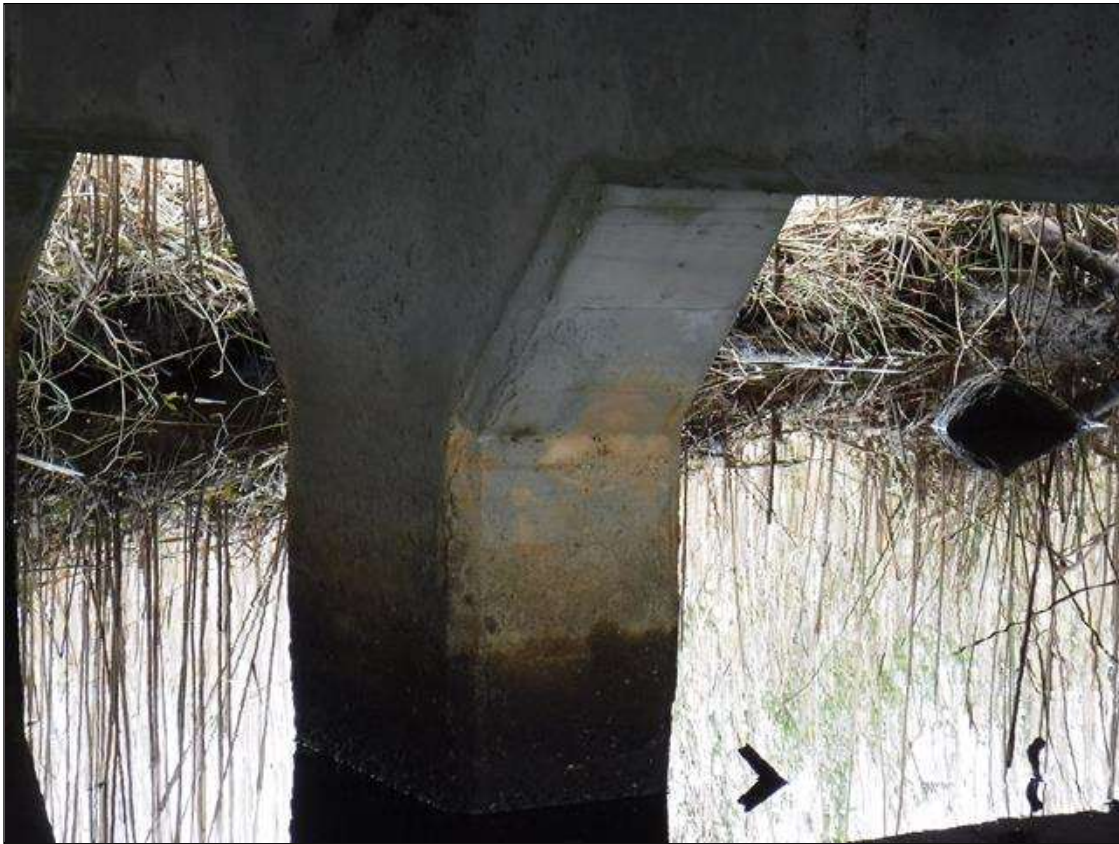
Bent 312 Pile 2: (2) 16" X 6" PATCHED AREAS, SOUTH FACE.
