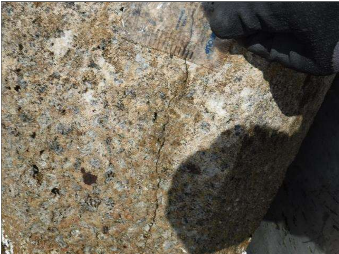
Bent 121 Pile 4: (PAR) UP TO 6' X 0.062" VERTICAL CRACKS, AT RANDOM THROUGHOUT.
