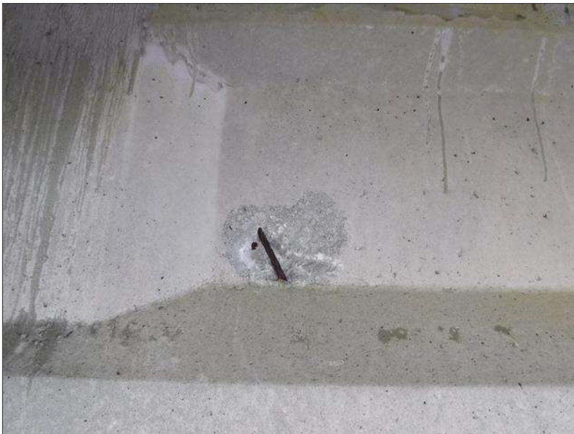
Span 130 Beam 2: (PAR) 9" X 6" X 1.5" DEEP SPALL, WITH EXPOSED STRAND, NORTH FACE, 3' FROM BENT 130.
