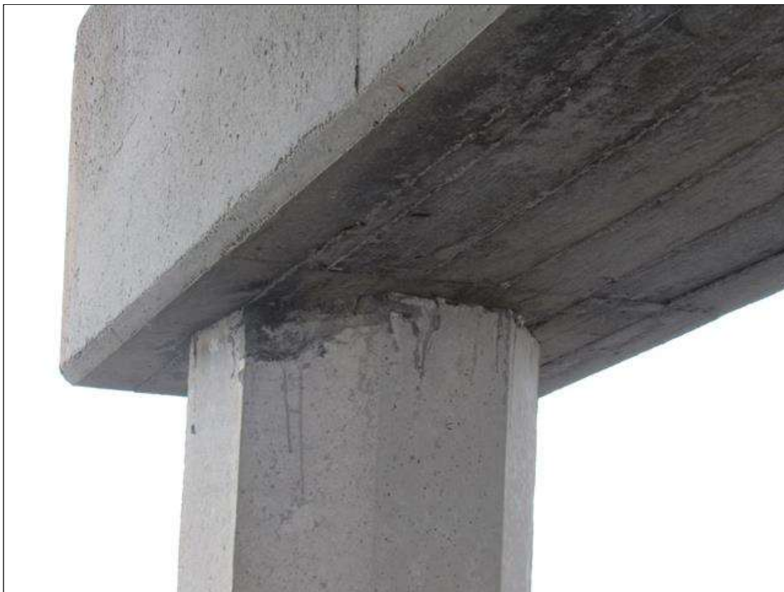
Bent 48 Saved Pile 1: 3" X 5" PATCHED AREA, SOUTH AND WEST FACES, AT BOTTOM OF CAP.
