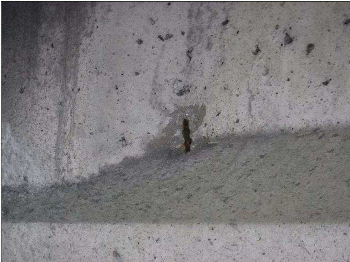
Span 206 Beam 3: 4" DIAMETER SPALL WITH EXPOSED REBAR IN WEB AT BENT 206
