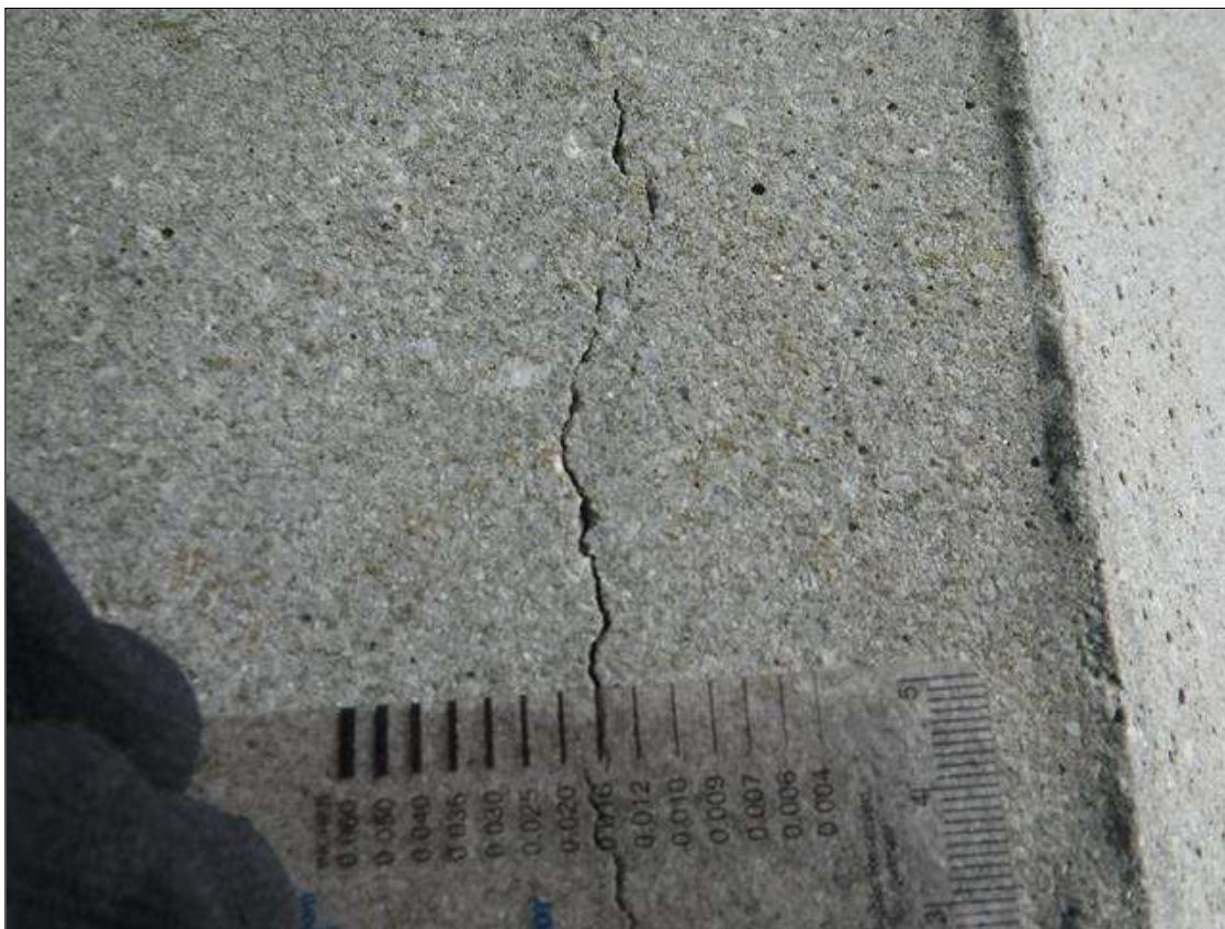
Bent 130 Pile 4: (PAR) UP TO 3' X 0.016" VERTICAL CRACKS, AT RANDOM THROUGHOUT.
