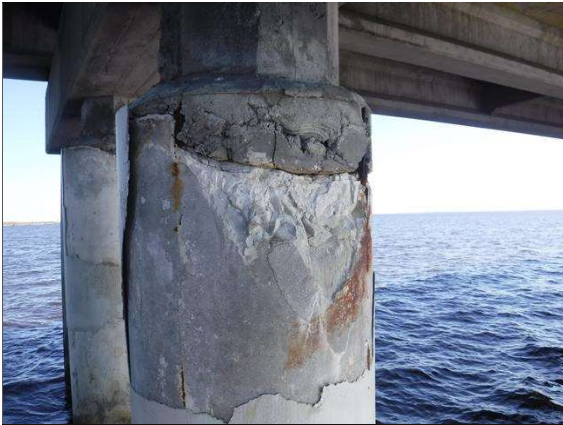
Bent 15 Saved Pile 3: (PAR) 10" X 2" UP TO 1" SPALL, SOUTH FACE, 2' FROM BOTTOM OF CAP, NORTH FACE SIMILAR
