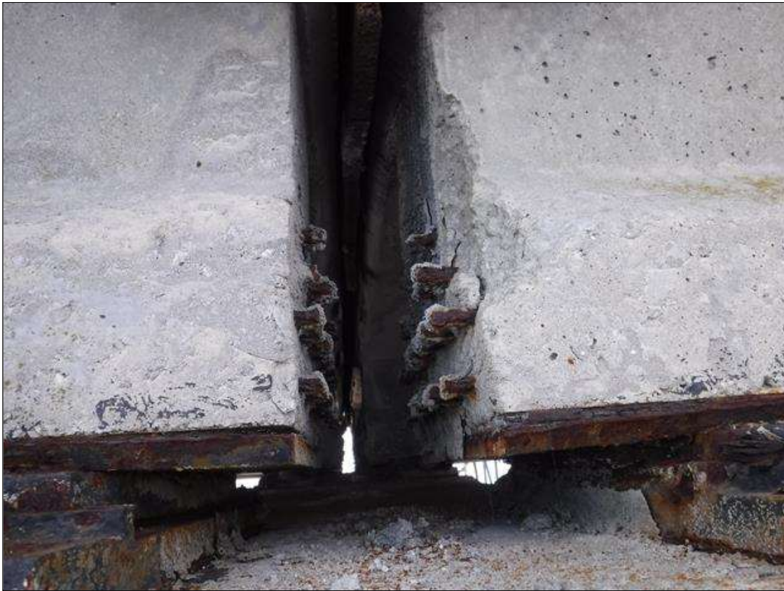
Span 81 Beam 1: 2" X 12" X 1" CORNER SPALL, NORTH FACE, AT BENT 81.
