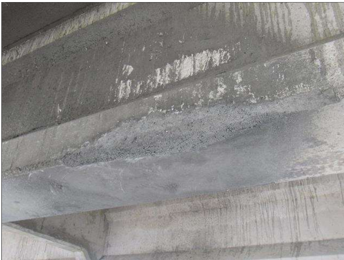
Span 45 Beam 2: 2.5' X UP TO 3" PATCHED AREA, BOTTOM FACE, EXTENDING 3" ONTO SOUTH FACE, 15' FROM BENT 45.
