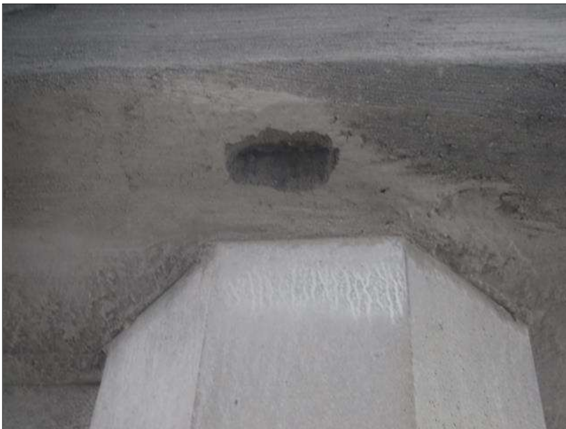
Bent 141 Cap 1: 6" DIAMETER X 2" DEEP SPALL WITH EXPOSED REBAR IN BOTTOM OF CAP EAST OF PILE 2
