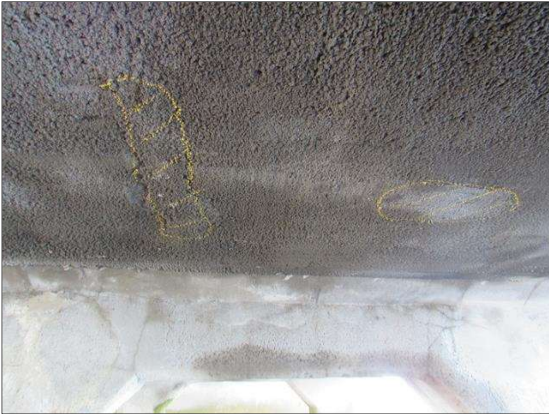
Span 280 Deck: (2) DELAMINATIONS UP TO 6" X 32" ON BOTTOM FACE LOCATED NEAR BENT 279 BETWEEN PILES 1 AND 2
