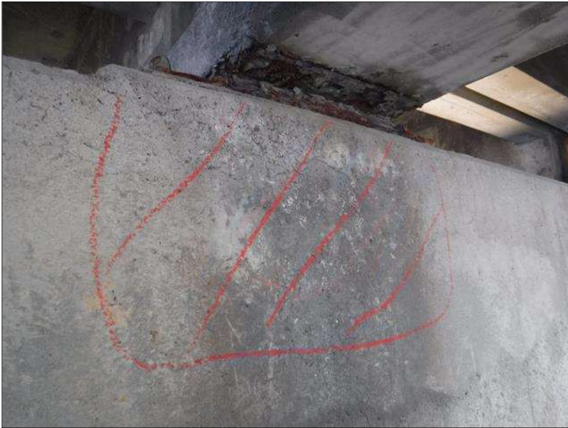
Bent 12 Cap 1: 16" X 12" DELAMINATION, TOP OF WEST FACE, BENEATH BEAM 2.
