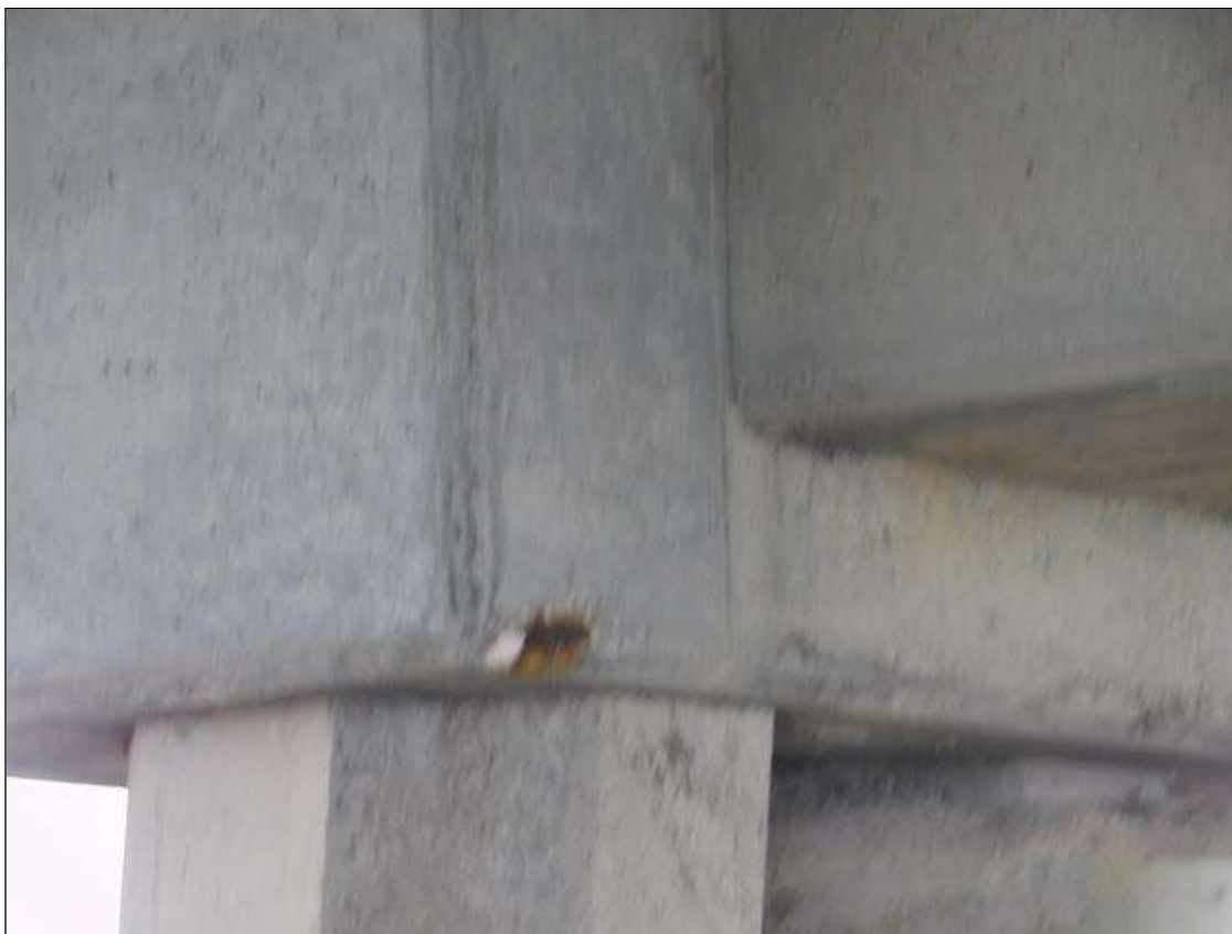
Bent 93 Cap 1: 8" X UP TO 3" X 2" SPALL, WITH EXPOSED REINFORCING, WEST FACE, TOP OF PILE 2.
