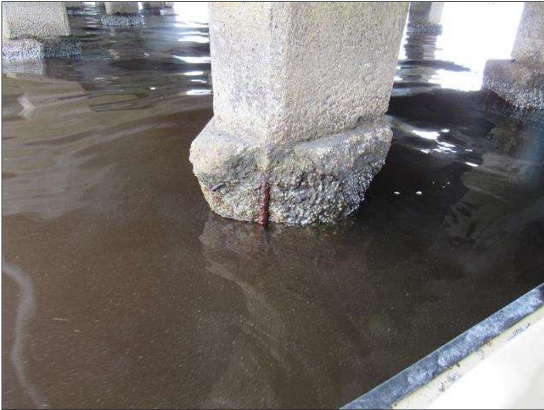
Bent 282 Pile 1: (PAR) 24" X UP TO 24" X 24" SPALL WITH EXPOSED REBAR AND COMPLETE SECTION LOSS TO VERTICAL BARS, WEST FACE OF COLUMN FOOTING.
