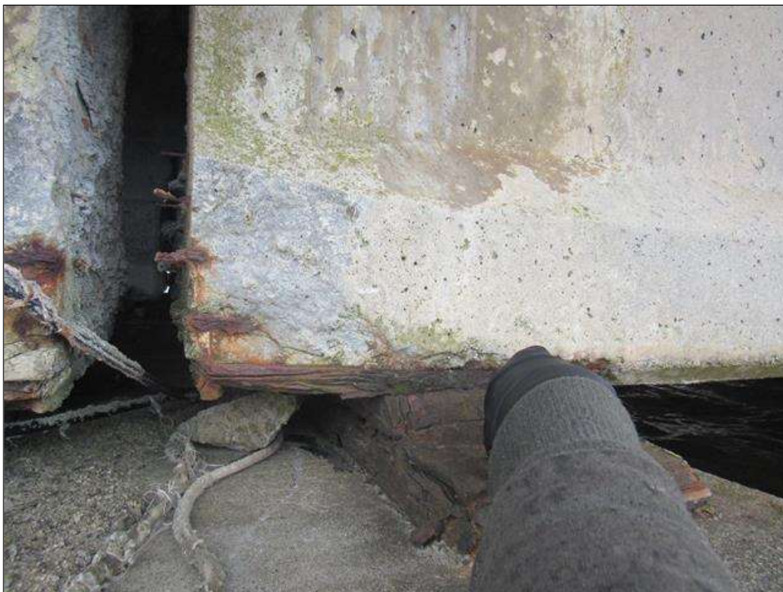
Span 1 Beam 1: (PAR) 8" x 8" x 2" DEEP SPALL (2) EXPOSED PRESTRESSED STRANDS ON RIGHT FACE LOCATED 8' FROM BENT 1
