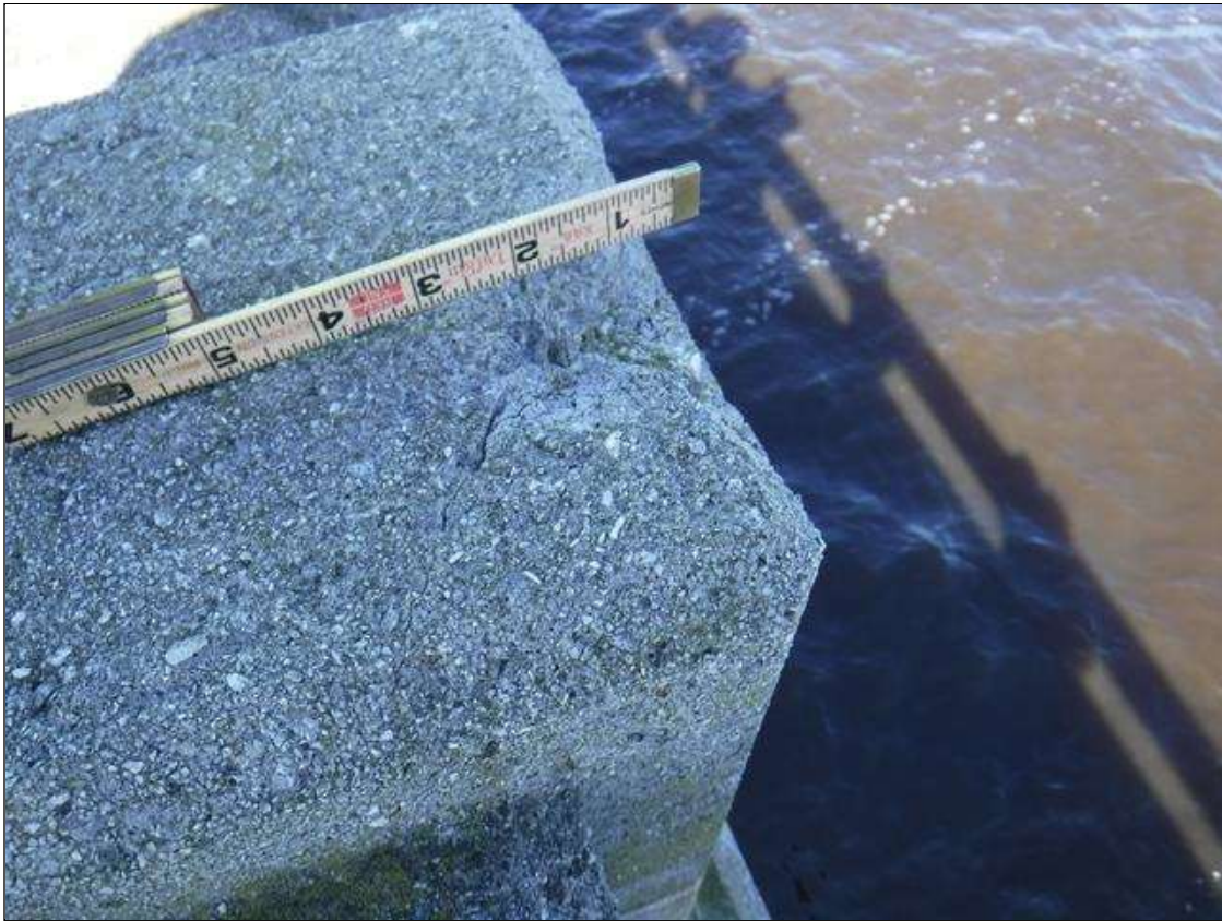
Span 18 Left Bridge Rail: 2 1/2" X 4" X 1 1/2" SPALL ON TOP FACE LOCATED FIRST POST AT BENT 17
