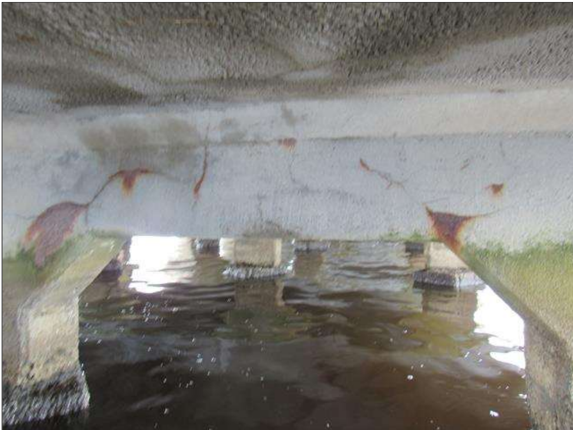
Bent 286 Cap 1: (PAR) 10' OF UP TO 1/16" WIDE TRANSVERSE AND LONGITUDINAL CRACKS WITH RUST STAINING, EAST FACE, BAY 1.
