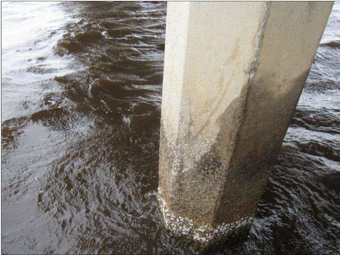
Bent 107 Pile 4: (PAR) (2) UP TO 3' X 0.02" VERTICAL CRACKS, SOUTH FACE, BEGINNING 9' FROM BOTTOM OF CAP, WITH ADJACENT 2' X UP TO 1' DELAMINATION.
