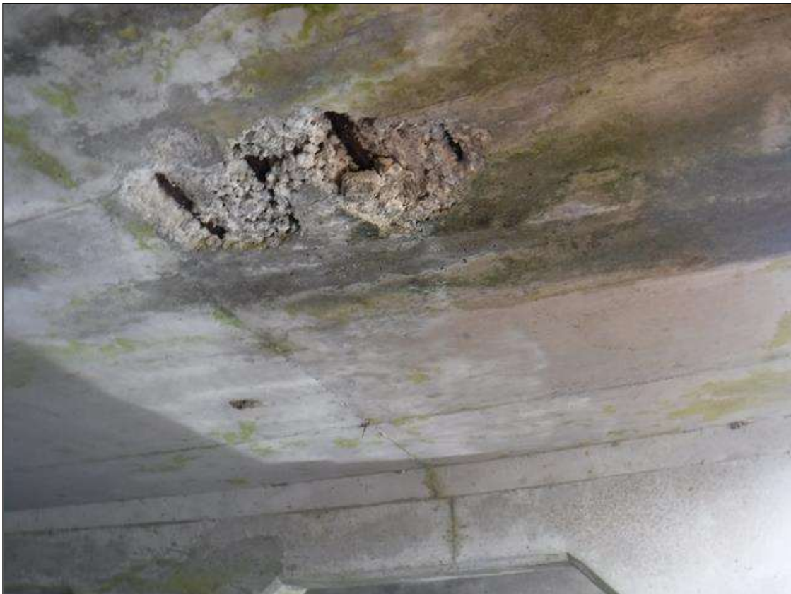
Span 309 Deck: (PAR) 20" X 10" X 1" SPALL WITH EXPOSED REBAR, DECK UNDERSIDE, 4' FROM SOUTH EDGE, NEAR MIDSPAN.
