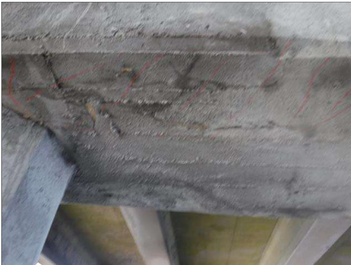
Bent 164 Cap 1: 4' X 1' DELAMINATION ON BOTTOM OF CAP BETWEEN PILES 2 AND 3
