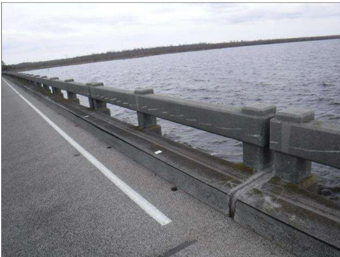
Span 259 Left Bridge Rail: 24' OF SCRAPES AND GAUGES CAUSED BY IMPACT DAMAGE ON LEFT FACE LOCATED ALONG RAIL
