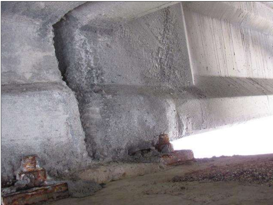
Span 57 Beam 2: (2) UP TO 24" X 12" PATCHED AREAS, NORTH AND SOUTH FACES, AT BENT 56.
