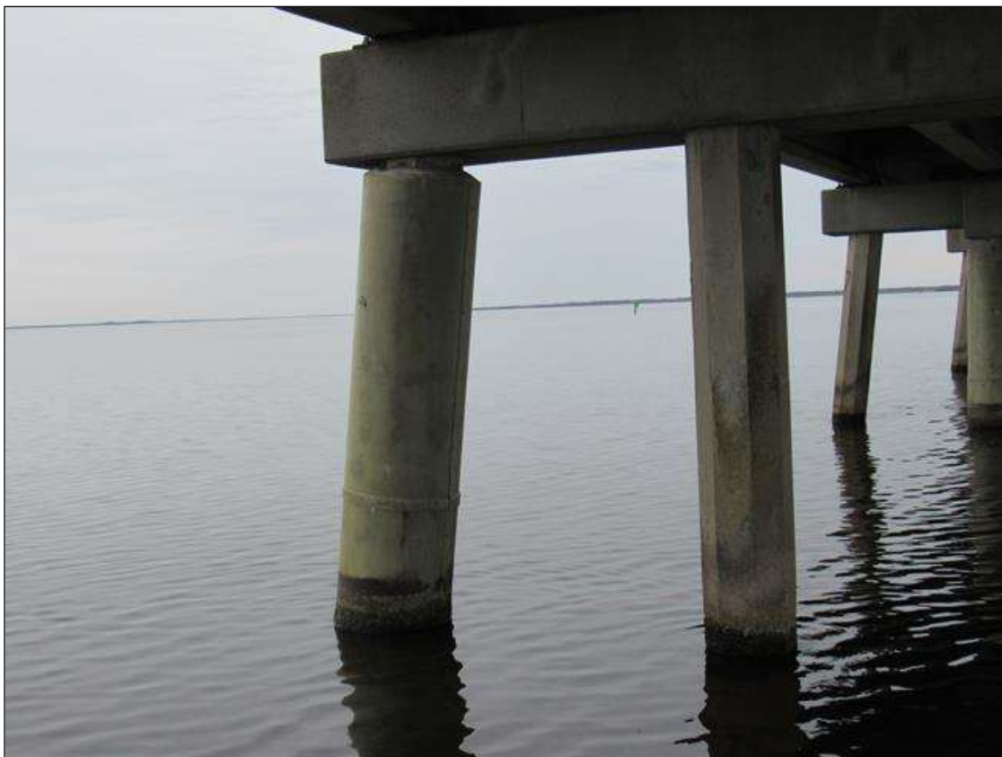
Bent 36 Saved Pile 1: PILE HAS BEEN JACKETED, BEGINNING 1' FROM BOTTOM OF CAP AND EXTENDING BELOW WATERLINE.
