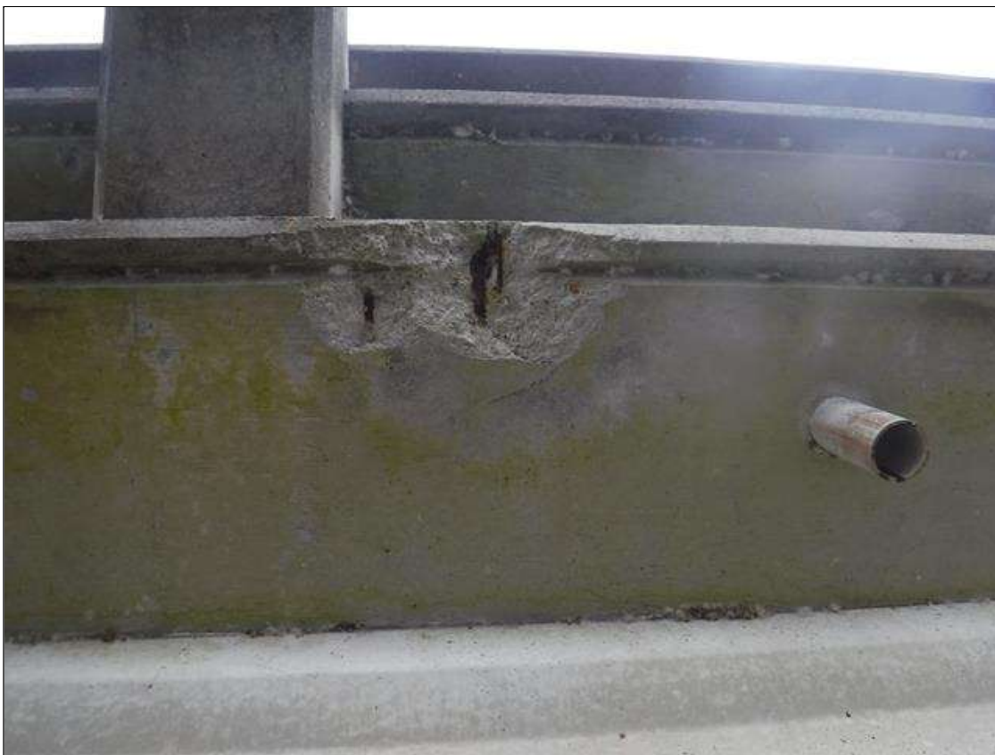
Span 242 Deck: (PAR) 2' X 1' X 2" DEEP SPALL IN DECK UNDERSIDE LEFT OVERHANG AT MIDSPAN
