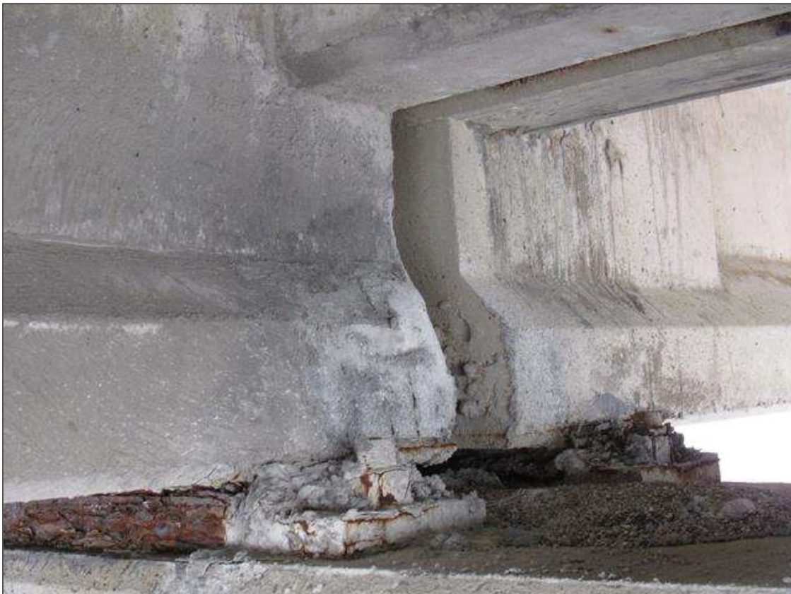
Span 68 Beam 2: (2) UP TO 18" X 18" PATCHED AREAS, NORTH AND SOUTH FACES, AT BENT 68.
