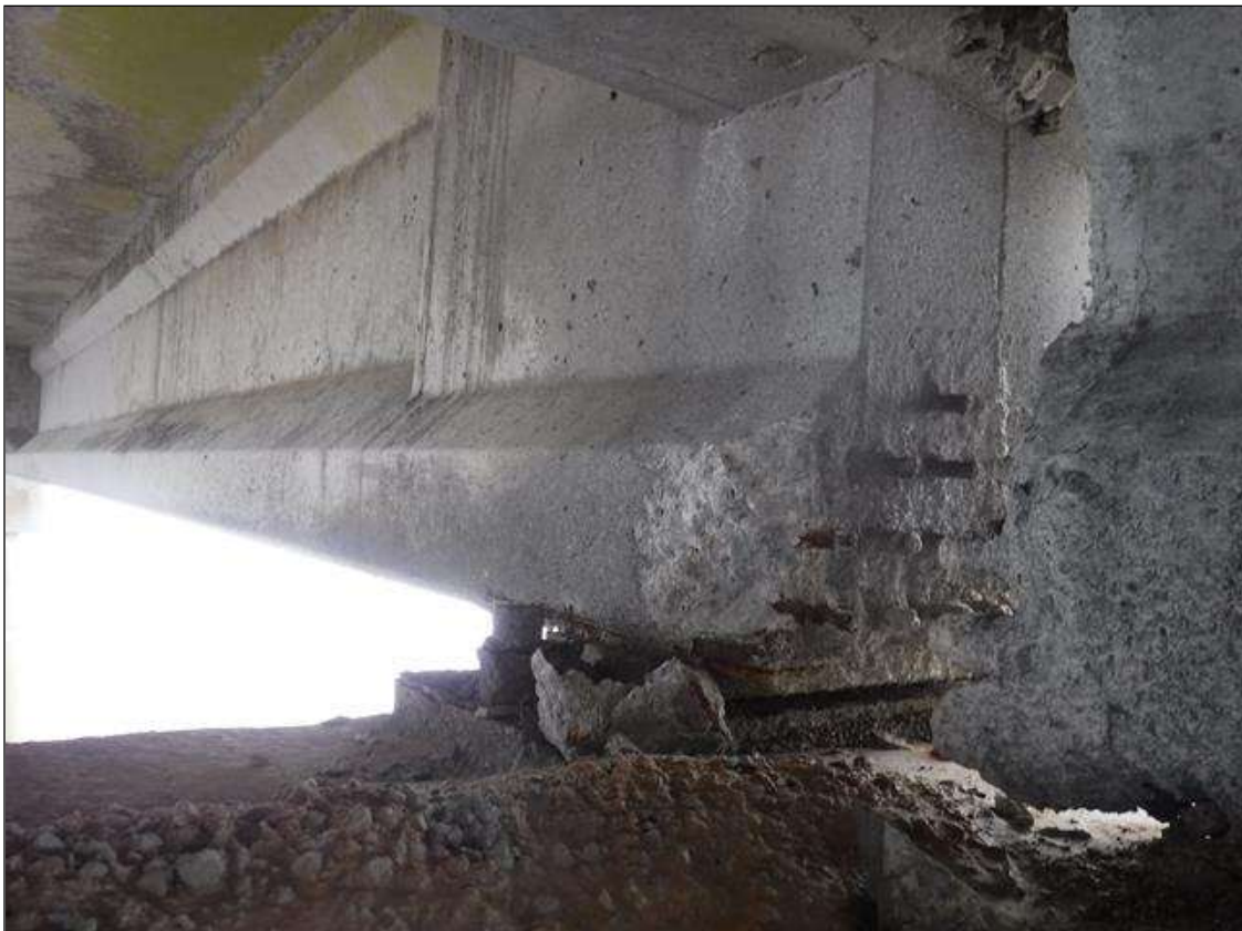
Span 90 Beam 4: (PAR) 6" X 6" X 2" DEEP SPALL WITH EXPOSED STRAND ON NORTH FACE AT BENT 89
