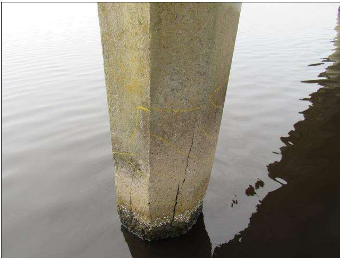
Bent 35 Saved Pile 1: 3' X 40" DELAMINATION, EAST AND WEST FACES, 8' FROM BOTTOM OF CAP.
