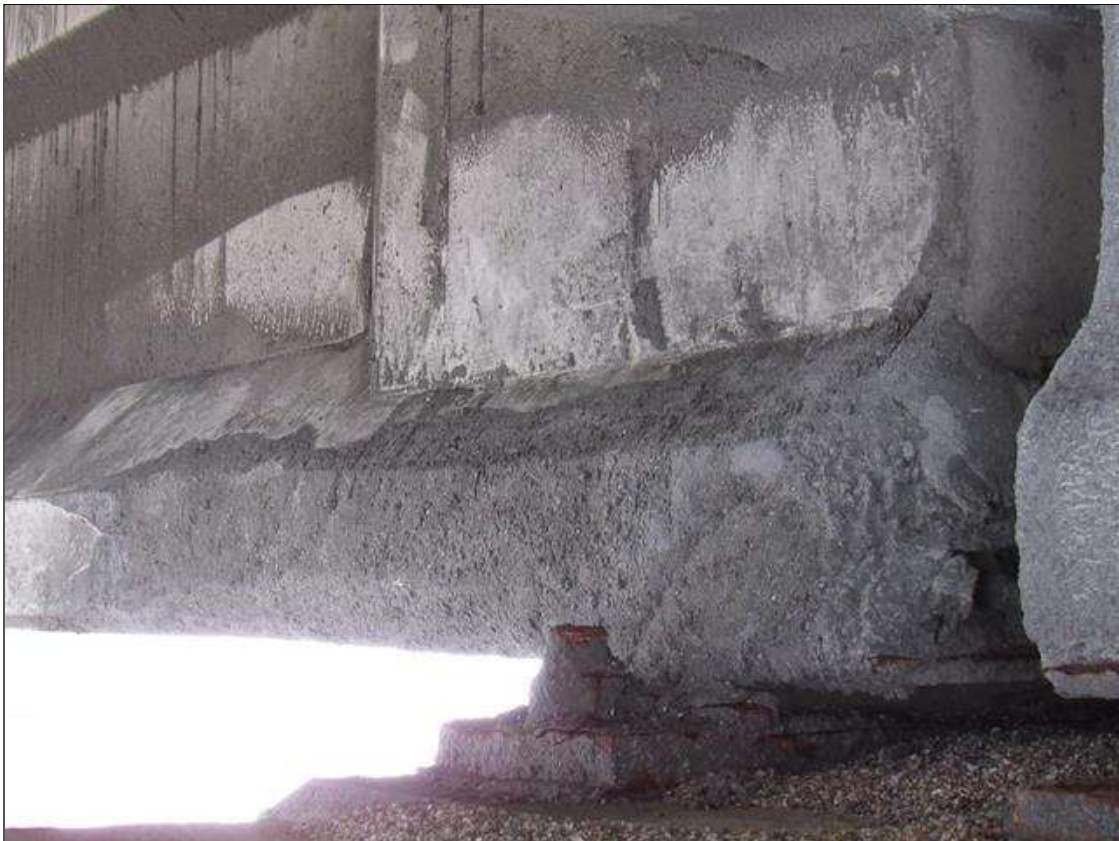
Span 47 Beam 2: 5' X UP TO 6" PATCHED AREA, BOTTOM FACE, EXTENDING 1' ONTO NORTH FACE, AT BENT 46.
