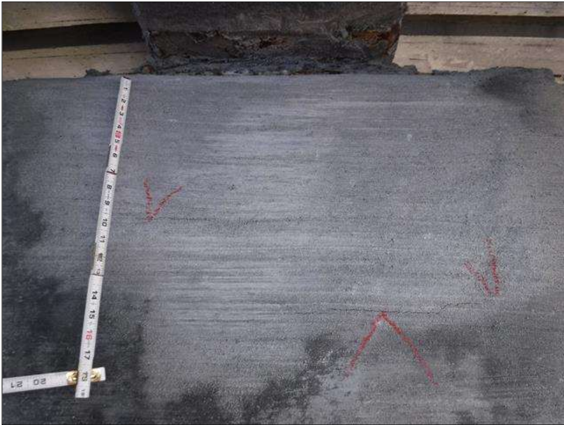
Bent 217 Cap 1: 2' PATCH WITH 1/32" CRACK BELOW BEAM 3 WEST FACE
