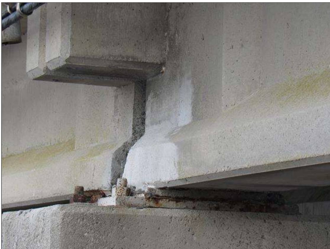
Span 32 Beam 4: 1' X 1' PATCHED AREA, NORTH AND SOUTH FACES, AT BENT 31.
