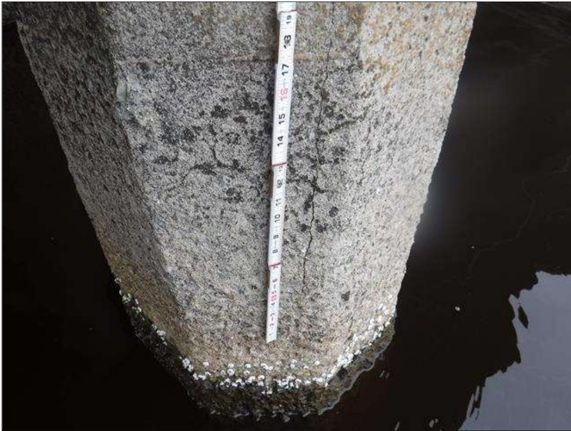
Bent 244 Pile 6: (PAR) (2) UP TO 2' X 0.03" VERTICAL CRACKS ON SOUTH FACE, BEGINNING 8' FROM BOTTOM OF CAP, AT RANDOM THROUGHOUT.
