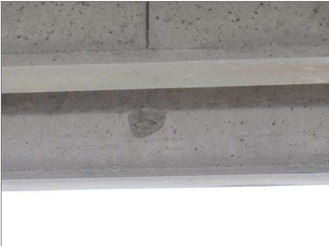
Span 51 Beam 1: 3" DIAMETER X 1" DEEP SPALL ON SOUTH FACE OF BOTTOM FLANGE LOCATED 15' FROM BENT 51
