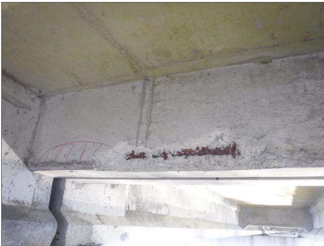
Span 127 Beam 3: (PAR) 5' X 1' X 2" DEEP SPALL WITH EXPOSED REBAR, WEST FACE OF BENT 127 DIAPHRAGM, BETWEEN BEAMS 3 AND 4
