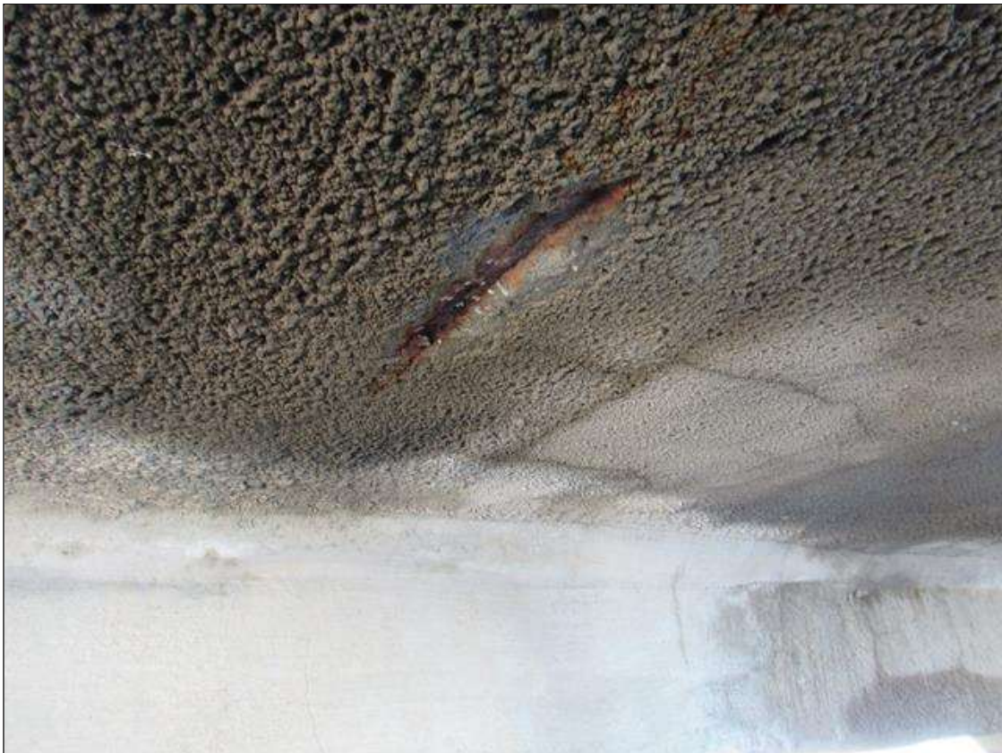
Span 281 Deck: (PAR) 3" X 12" X 1/2" DEEP SPALL WITH EXPOSED REBAR ON BOTTOM FACE LOCATED NEAR BENT 280, PILE 2
