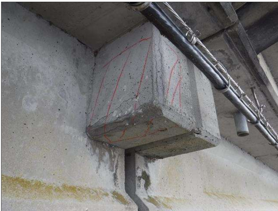
Span 91 Beam 4: 1' X 1' DELAMINATION, END DIAPHRAGM, RIGHT OVERHANG, AT BENT 91.
