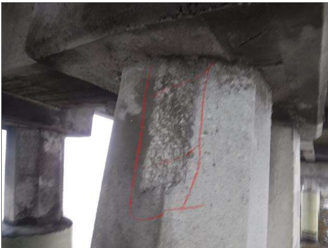
Bent 195 Pile 4: 16" X 6" X 1" SPALL, WEST FACE, AT BOTTOM OF CAP.
