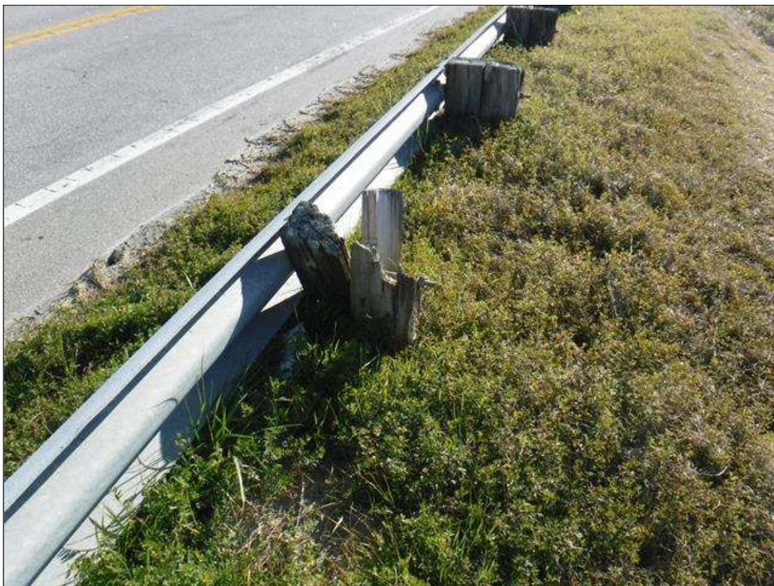
(PAR) BROKEN POST ON NEAR RIGHT GUARDRAIL 75' FROM END BENT 1
