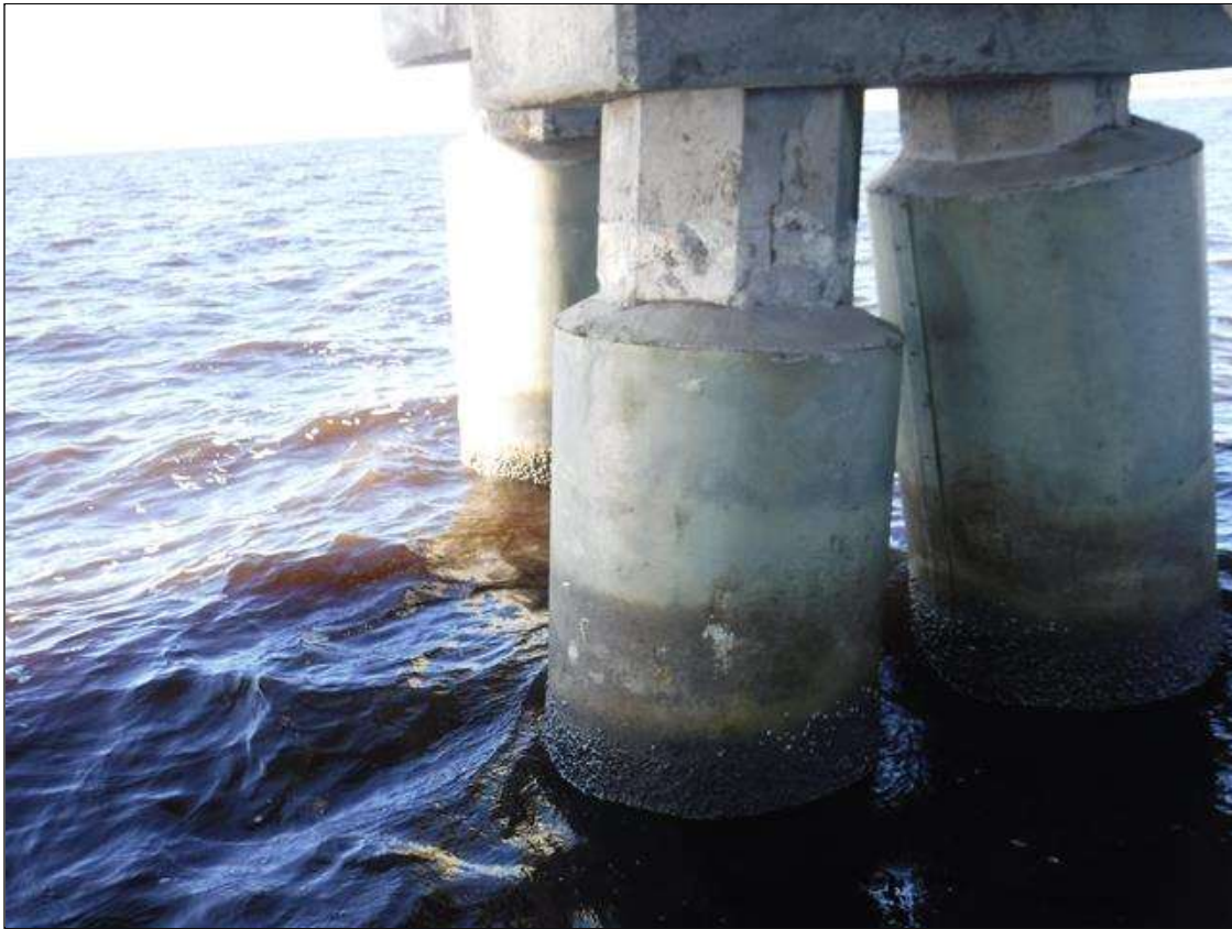
Bent 9 Saved Pile 5: PILE REPAIRED WITH 3' DIAMETER CONCRETE JACKET STARTING 18" BELOW BOTTOM OF CAP, TYPICAL REPAIR METHOD TO MULTIPLE PILES THROUGHOUT BRIDGE.
