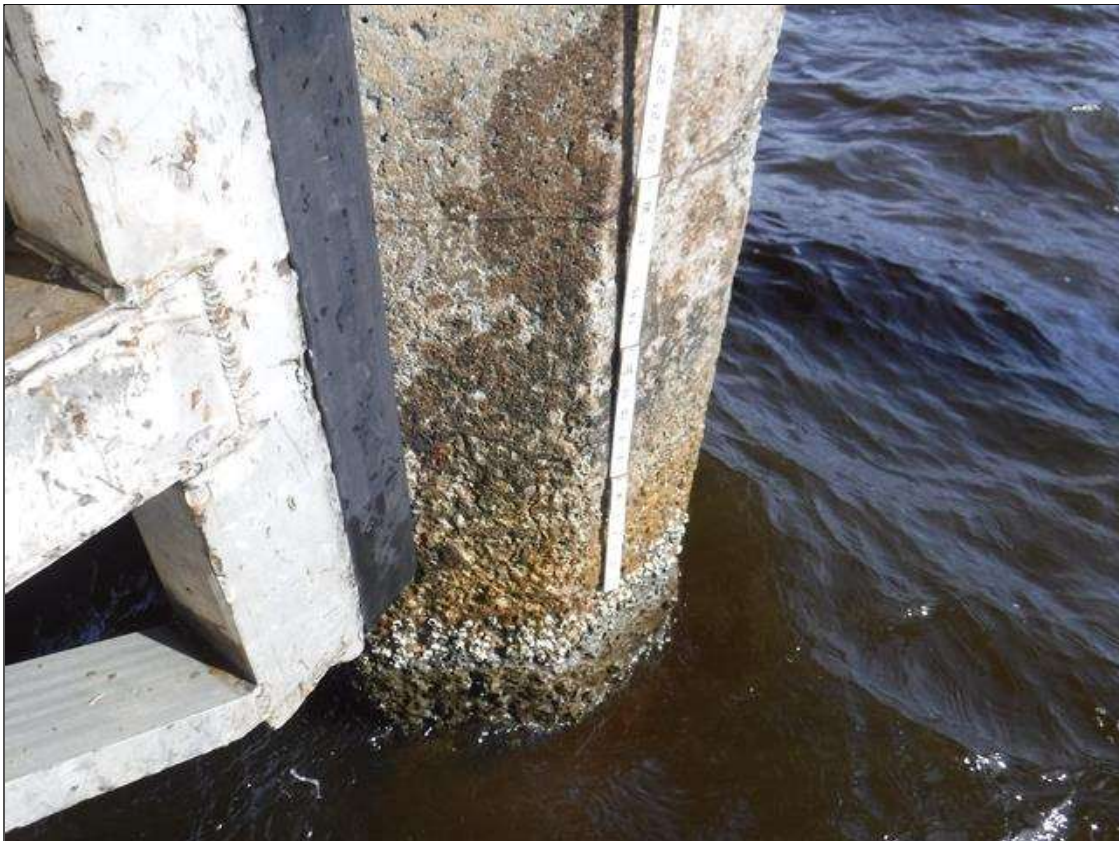
Bent 124 Pile 3: (2) 3' X 1' DELAMINATIONS, NORTH AND WEST FACES, 7' FROM BOTTOM OF CAP, EXTENDING BELOW WATERLINE.
