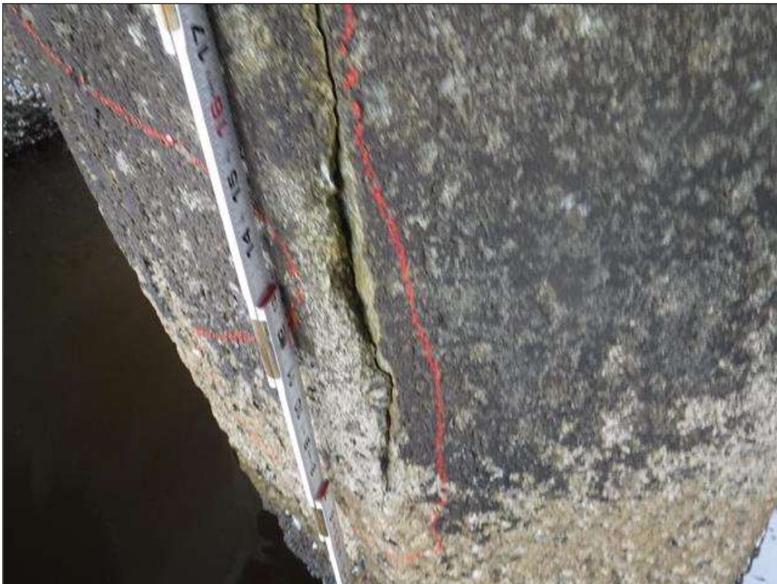
Bent 243 Pile 4: (PAR) HAIRLINE TO 1/4" CRACKS, 8' BELOW CAP, DOWN 4' , MULTIPLE FACES. SCALING TO 1" DEEP WITH LOOSE AGGREGATE FROM WATERLINE TO MUDLINE.
