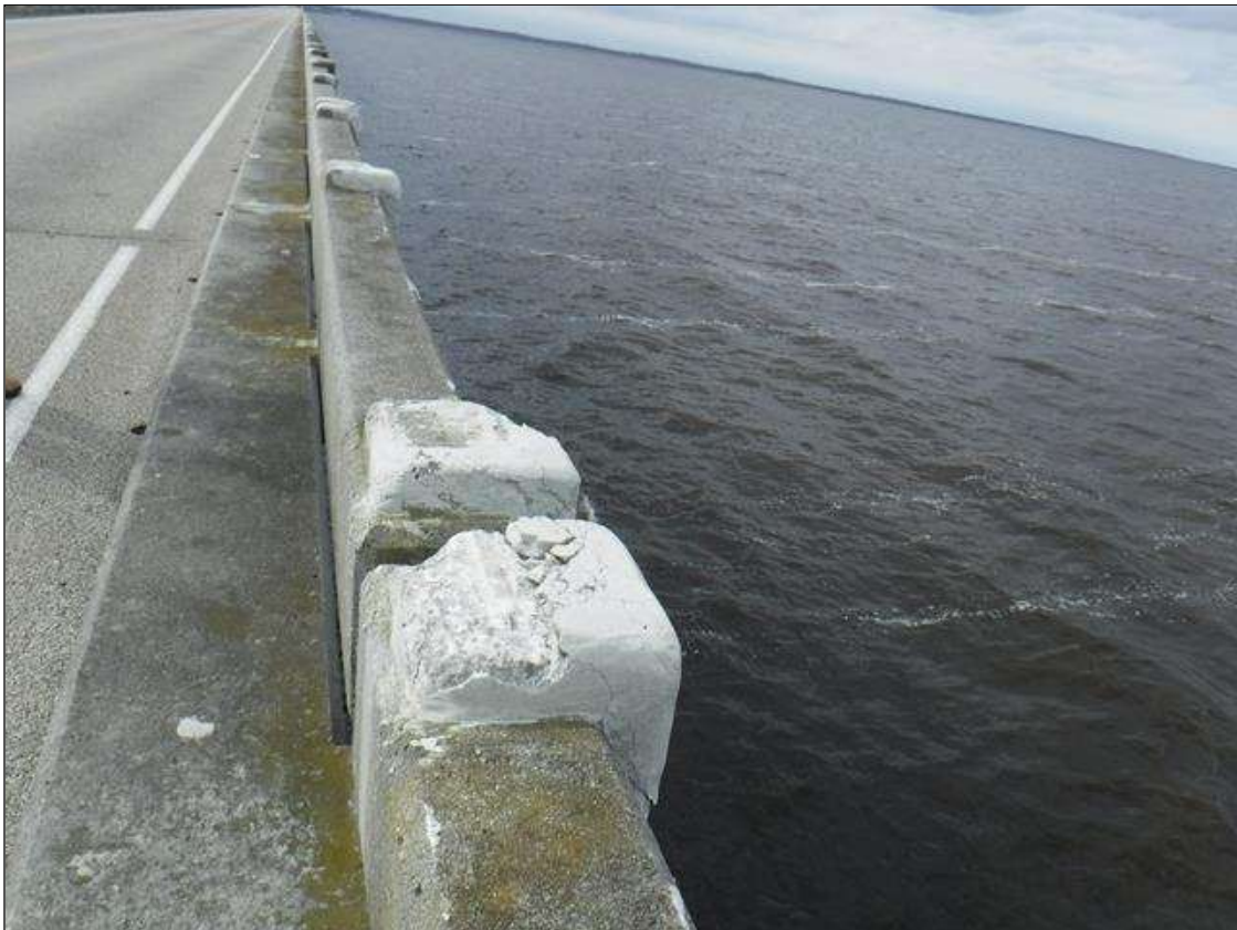
Span 242 Left Bridge Rail: (8) UP TO 10" X 10" CRACKED PATCHED AREAS, WITH UP TO 6" X 6" X 4" SPALLS, SOME WITH EXPOSED REINFORCING, AT RANDOM THROUGHOUT TOP OF RAIL POSTS.
