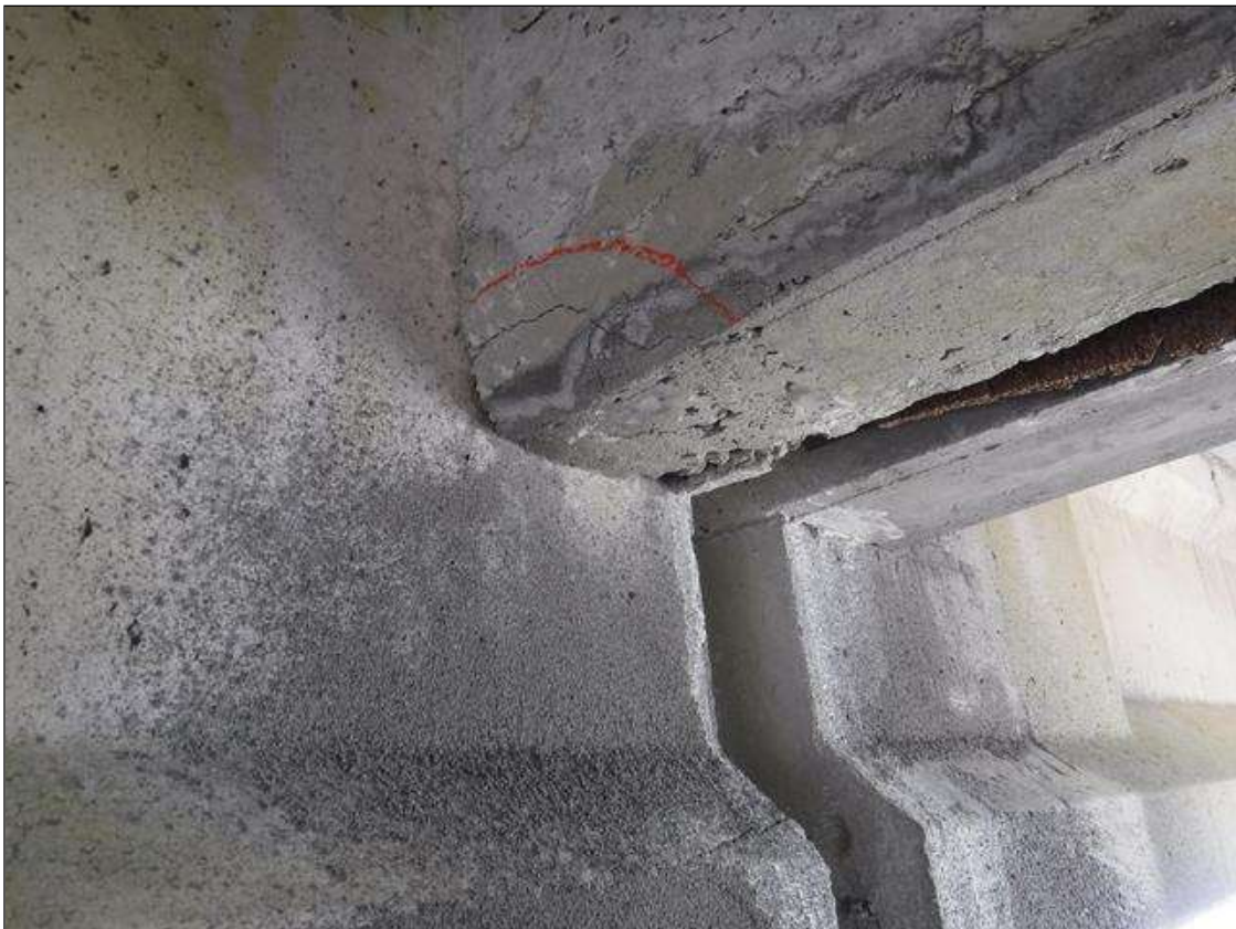
Span 83 Beam 2: 6" X 4" DELAMINATION IN BAY 2 DIAPHRAGM AT BENT 83
