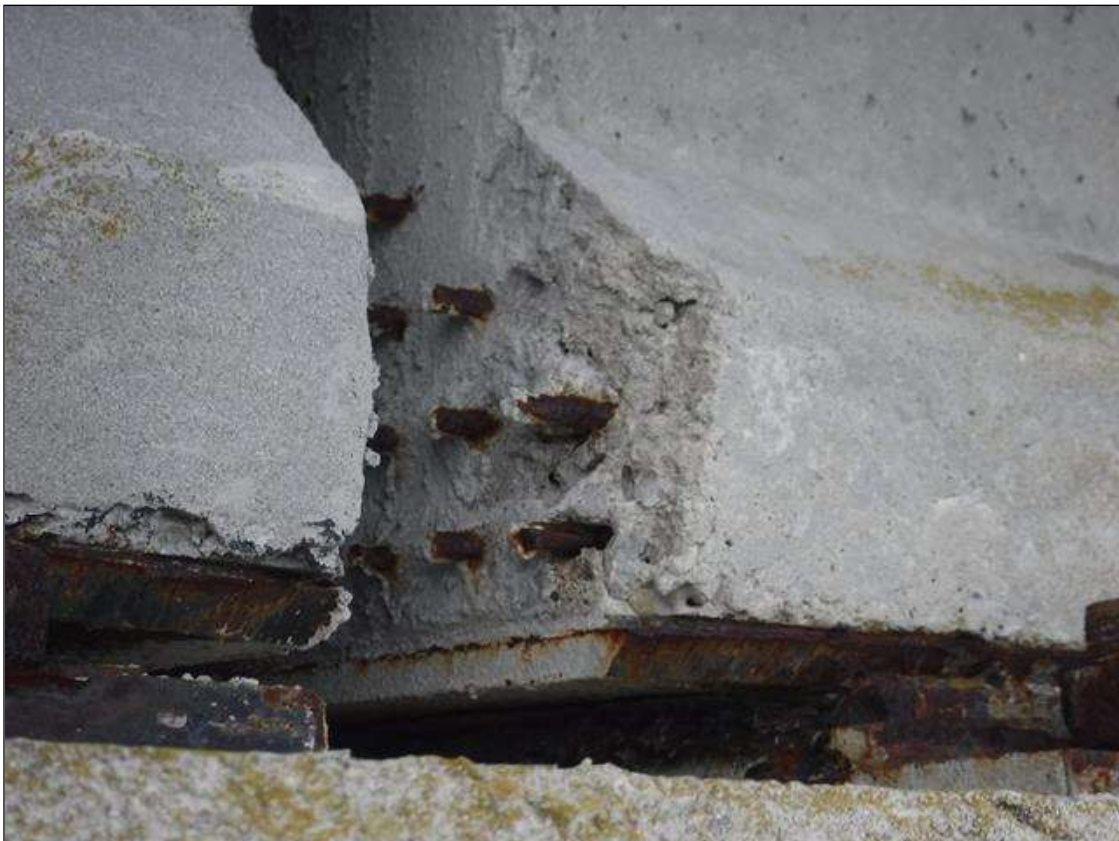
Span 179 Beam 1: (PAR) 6" X 6" SPALL WITH EXPOSED STRAND, NORTH FACE, AT BENT 178.
