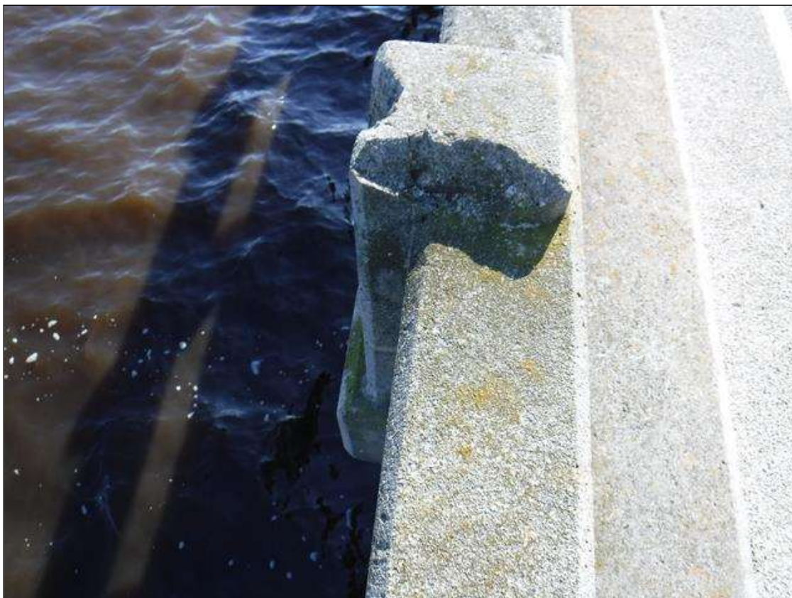
Span 2 Left Bridge Rail: 8" X 8" X UP TO 3" SPALL, WITH EXPOSED REINFORCING, NORTHWEST CORNER, 8TH RAIL POST FROM BENT 1.
