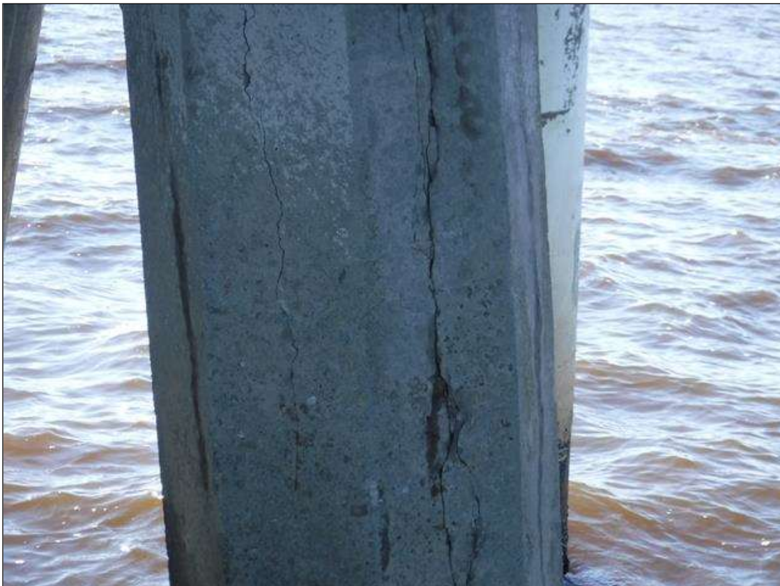
Bent 13 Saved Pile 4: (PAR) HAIRLINE TO 1/8" CRACKS, FROM BOTTOM OF CAP DOWN 8', MULTIPLE FACES. SCALING TO 1" DEEP FROM WATERLINE TO MUDLINE.
