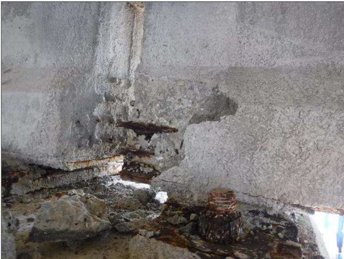
Span 145 Beam 4: (PAR) 6" X 10" X 2" DEEP SPALL WITH EXPOSED STRAND ON NORTH FACE AT BENT 145
