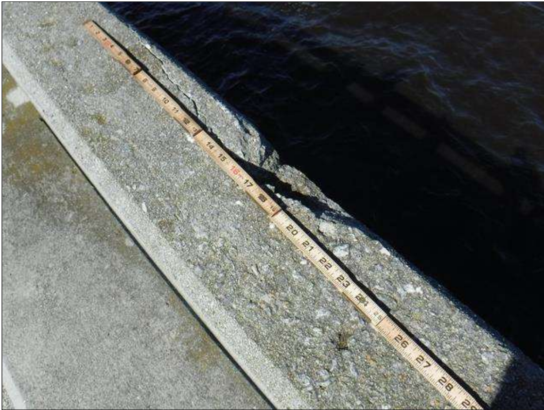
Span 100 Left Bridge Rail: 2' x 3" x 2" DEEP SPALL WITH DELAMINATION, TOP NORTH CORNER, 3' FROM BENT 100.
