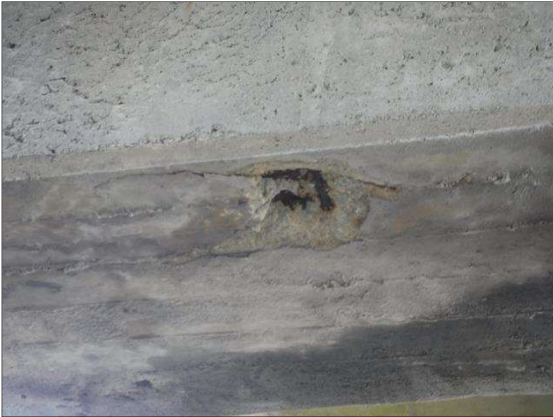
Bent 169 Cap 1: (PAR) 10" X UP TO 10" X 1.5" DEEP SPALL, WITH EXPOSED PRIMARY REINFORCING, BOTTOM OF CAP, BETWEEN COLUMNS 1 AND 2, WITH ADJACENT 6' X 10" DELAMINATION. REINFORCEMENT HAS 10% SECTION LOSS
