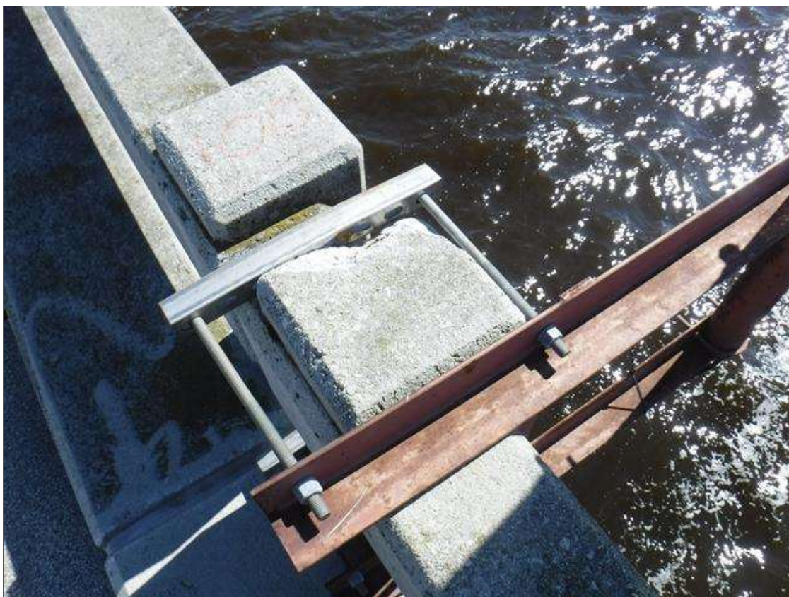
Span 99 Right Bridge Rail: 3" X 10" X UP TO 3" SPALL, WITH EXPOSED REINFORCING, TOP OF RAIL POST AT BENT 99.
