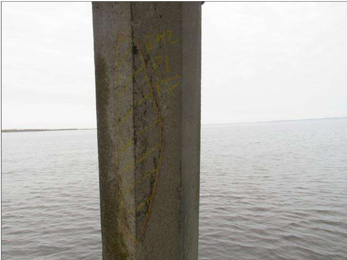
Bent 42 Saved Pile 2: 38" X 9" WIDE DELAMINATION ON SOUTH FACE 22" FROM BOTTOM OF CAP
