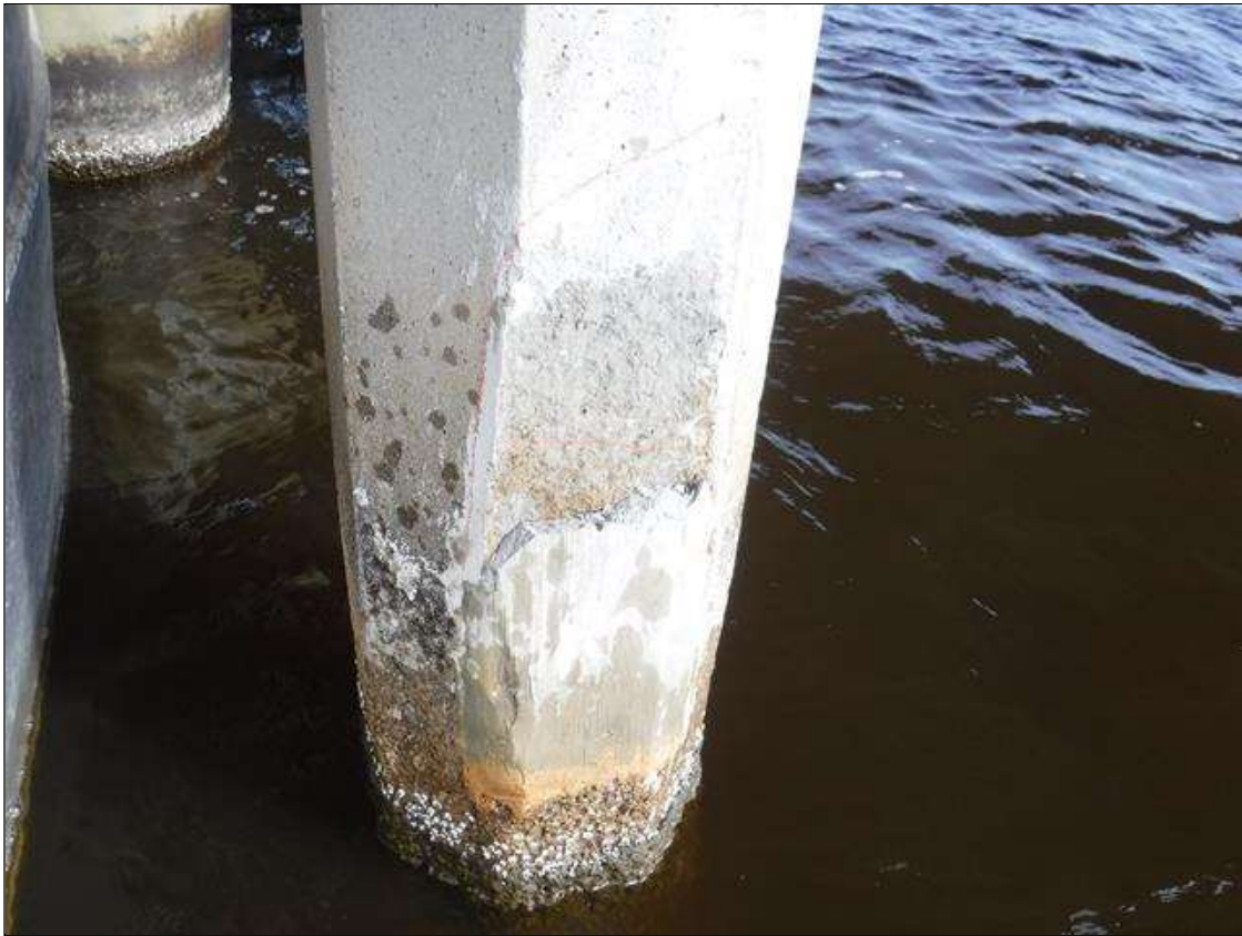
Bent 223 Pile 6: (PAR) 4' X UP TO 16" FAILED PATCH ON SOUTH FACE, 7' FROM BOTTOM OF CAP.
