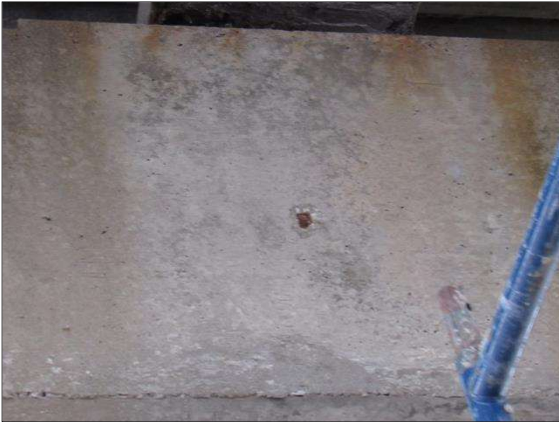
Bent 56 Cap 1: 2" DIAMETER SPALL WITH EXPOSED REINFORCING, EAST FACE, BENEATH BEAM 3.
