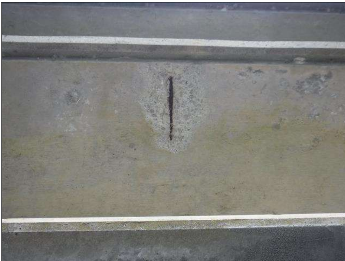
Span 236 Deck: (PAR) 16" DIAMETER X 1" DEEP SPALL WITH EXPOSED REINFORCEMENT IN DECK UNDERSIDE RIGHT OVERHANG, 15' FROM BENT 235
