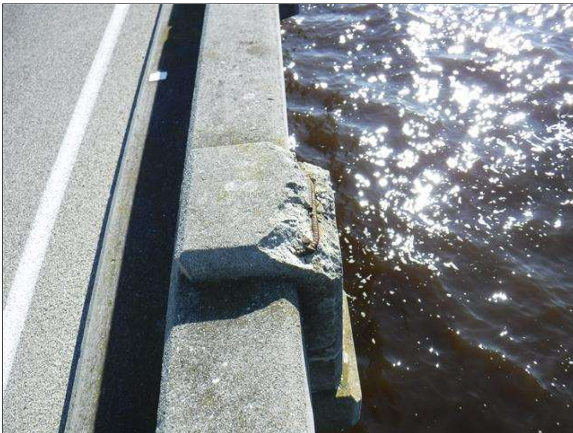
Span 8 Right Bridge Rail: 10" X 3" X UP TO 3" SPALL, WITH EXPOSED REINFORCING, SOUTH CORNER, 2ND RAIL POST FROM BENT 7.
