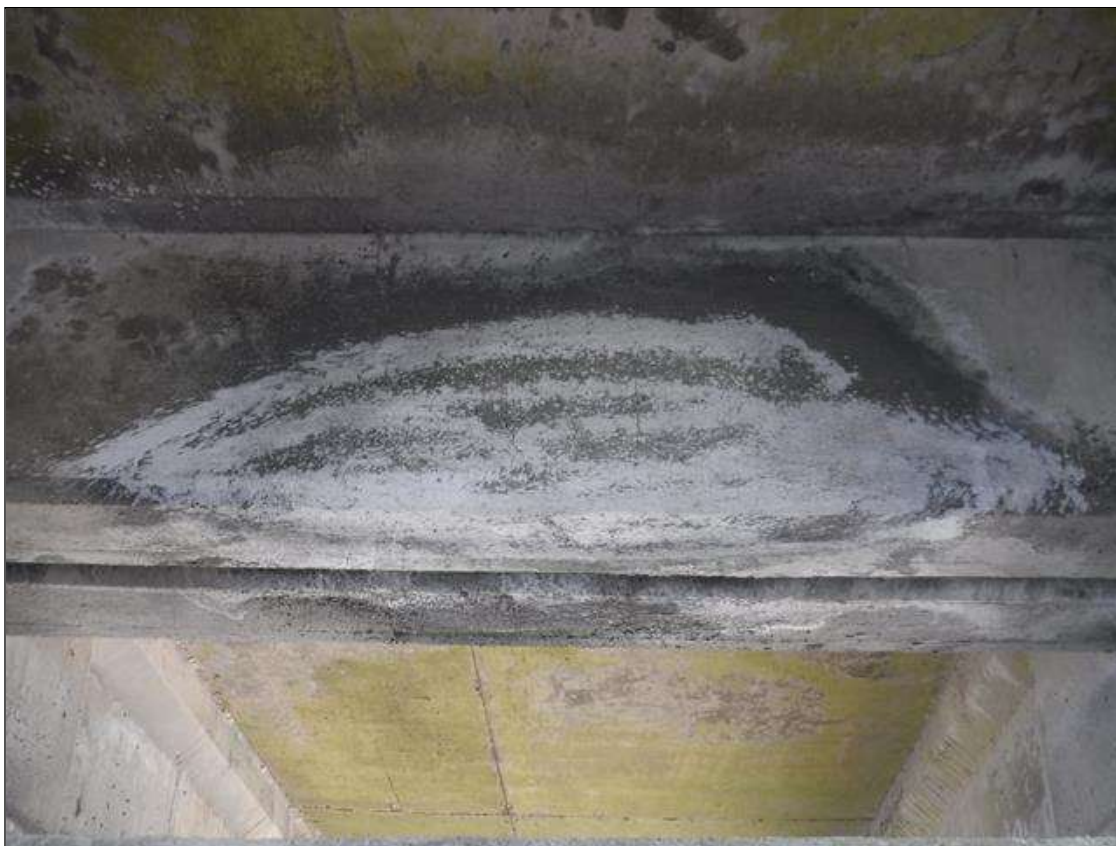
Span 152 Beam 3: 5' X UP TO 1' X 10" CRACKED PATCHED AREA UP TO 1/16", END DIAPHRAGM, BETWEEN BEAMS 3 AND 4, AT BENT 152.
