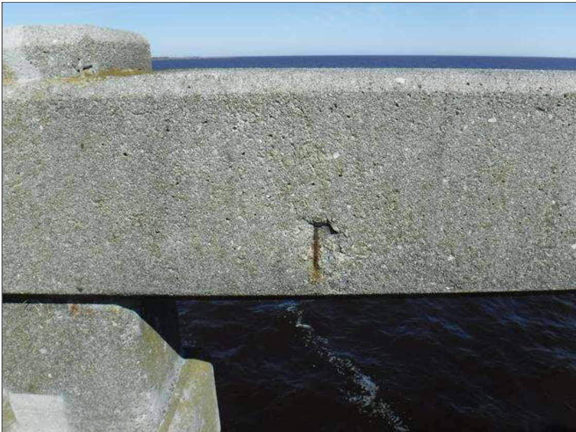
Span 67 Left Bridge Rail: 3" X 2" X 1/2" SPALL WITH EXPOSED REBAR ON RIGHT FACE LOCATED 1' PAST POST 4
