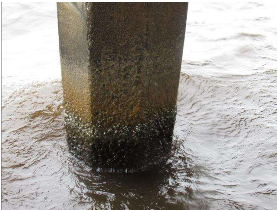
Bent 77 Pile 1: (PAR) (3) UP TO 2' X 0.03" VERTICAL CRACKS, BEGINNING 10' BOTTOM OF CAP, AT RANDOM THROUGHOUT.
