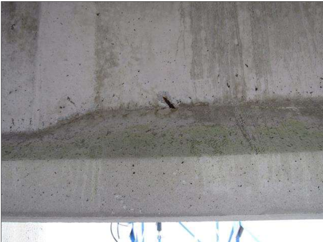
Span 54 Beam 4: (1) LOCATION OF EXPOSED REBAR, NORTH FACE, 5' FROM BENT 54.
