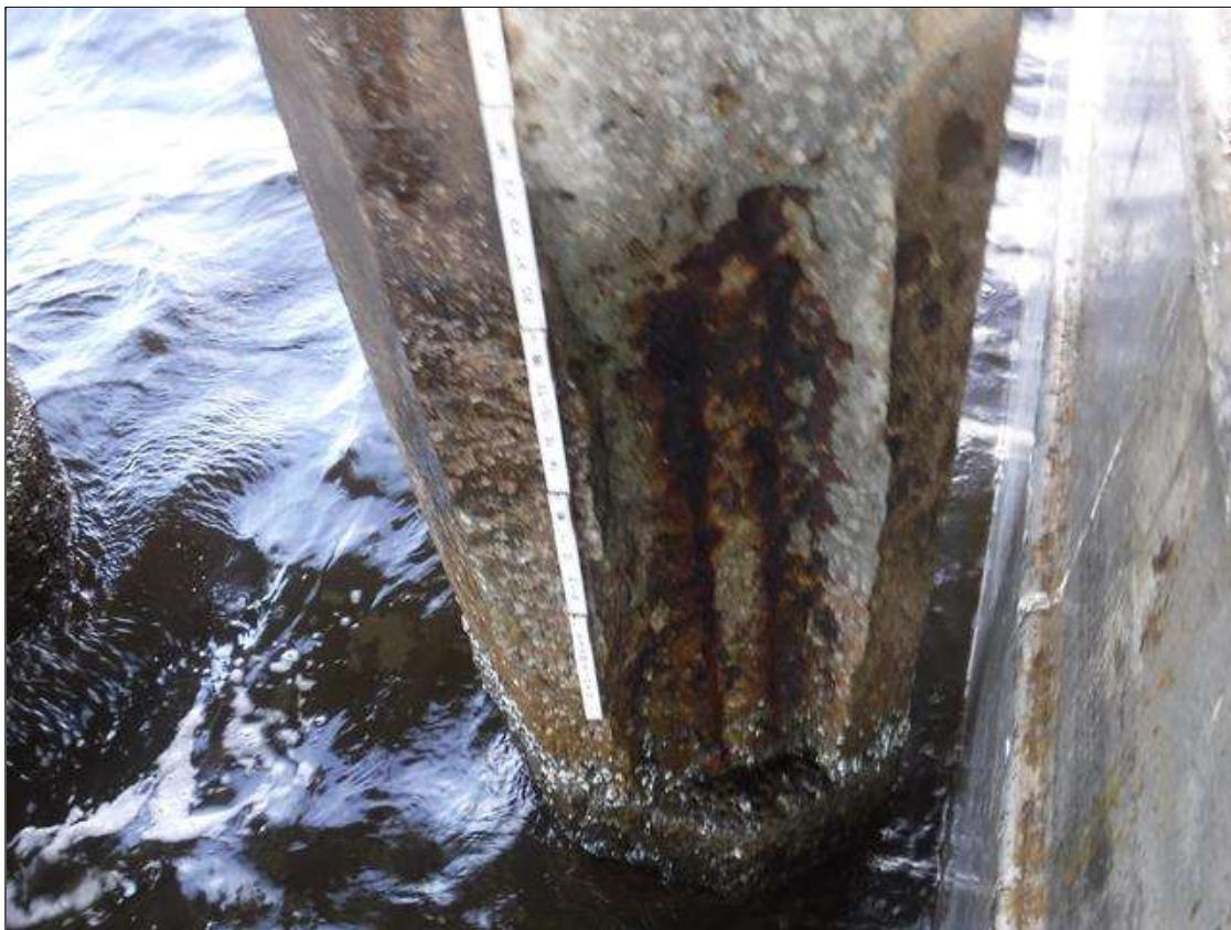
Bent 159 Pile 3: (PAR) 6' X UP TO 1' X 2.5" SPALL, WITH EXPOSED STRAND, SOUTH FACE, STARTING 4' FROM BOTTOM OF CAP.
