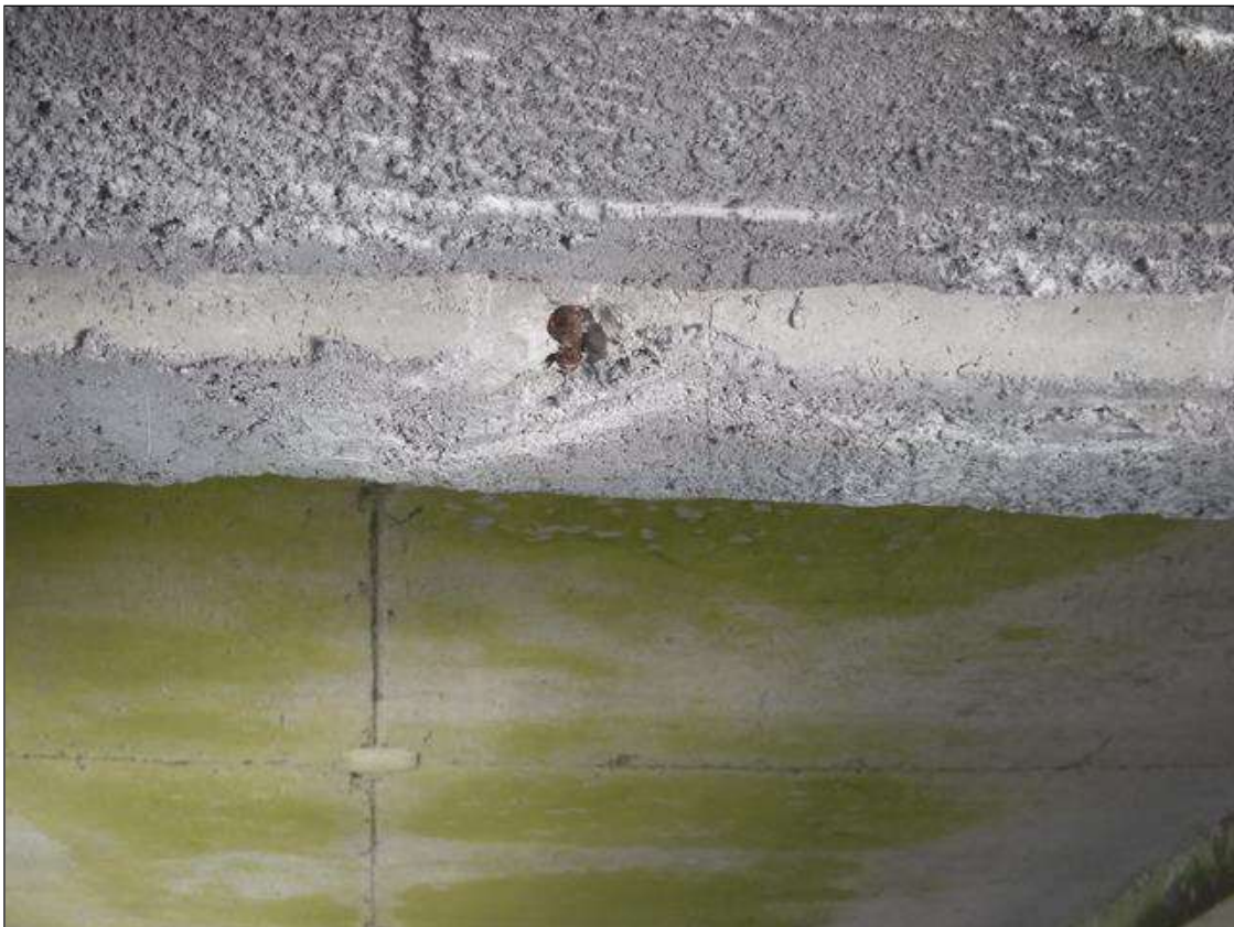
Span 115 Beam 3: 3' X UP TO 1' PATCHED AREA WITH 6" AREA OF EXPOSED REBAR, WEST FACE OF BENT 114 DIAPHRAGM, BETWEEN BEAMS 3 AND 4.
