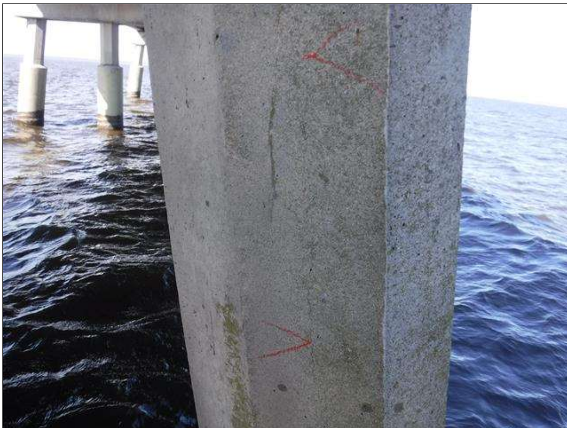
Bent 162 Pile 1: 10' LONG X 0.006" WIDE VERTICAL CRACK ON EAST FACE
