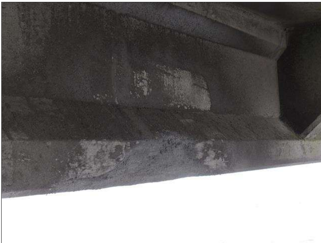
Span 41 Beam 4: 2.5' X UP TO 5" PATCHED AREA, BOTTOM FACE, EXTENDING 7" ONTO NORTH FACE, 18' FROM BENT 41.
