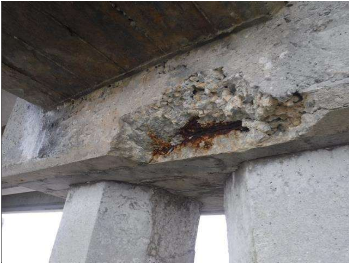
Bent 167 Cap 1: (PAR) 6" DEEP X UP TO 8" X 22" SPALL, WITH EXPOSED REINFORCING, BOTTOM OF CAP, NORTH OF PILES 2 AND 3. REBAR HAS 10% SECTION LOSS
