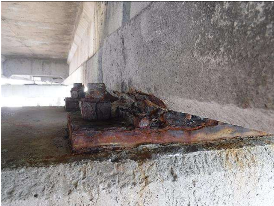
Span 73 Beam 4 Far Bearing: CORROSION WITH LESS THAN 1/16" LOSS. (2" REMAINING).
