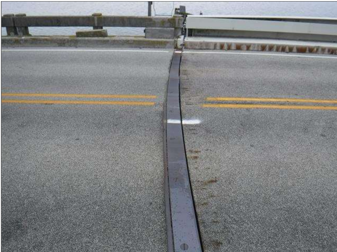
Expansion Joint 115 : NEW CONCRETE OVERLAY SINCE 2018 INSPECTION
