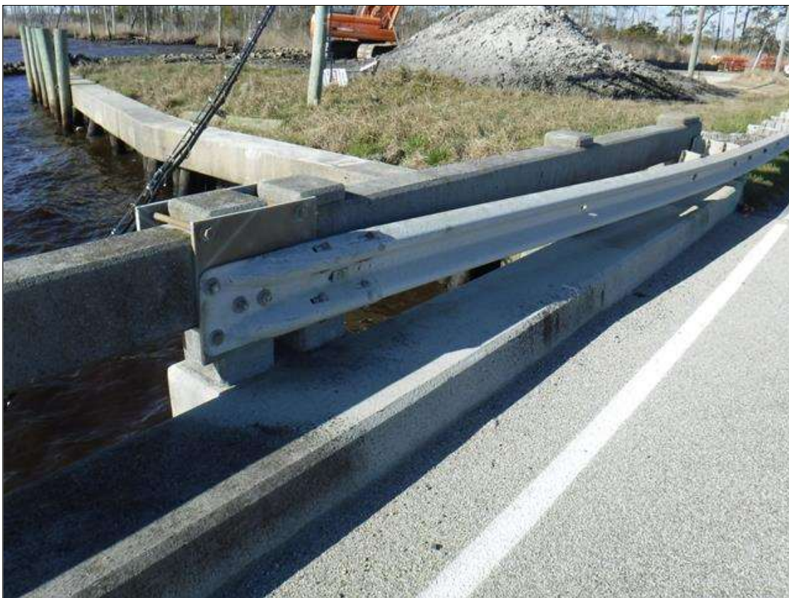
NEAR RIGHT GUARDRAIL ATTACHMENT
