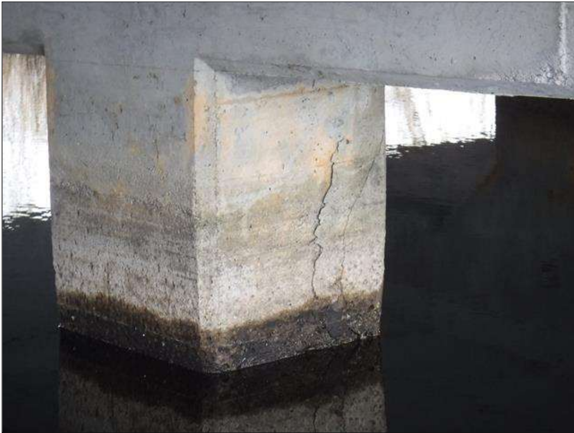
Bent 337 Pile 3: 24" X 12" X 10" DELAMINATION AT BOTTOM SOUTH CORNER
