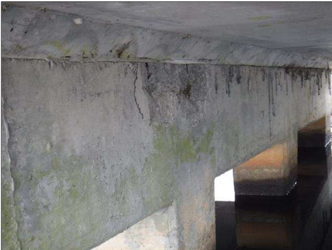
Bent 313 Cap 1: 30" X 12" X 2" SPALL, EAST FACE, ABOVE PILE 3.
