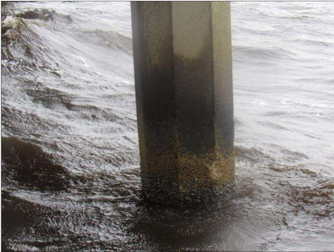
Bent 64 Pile 1: 6" X 4" X 1" SPALL, EAST FACE, 8' FROM BOTTOM OF CAP.
