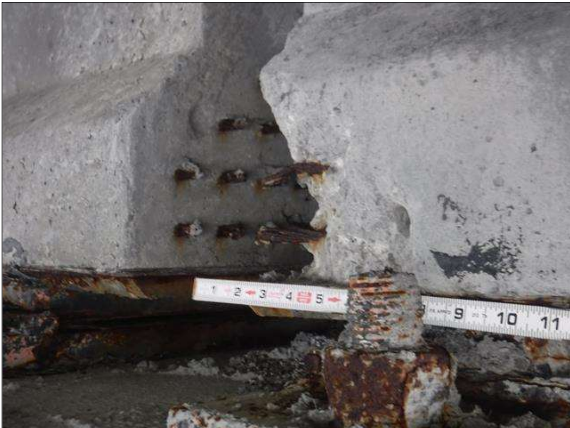
Span 237 Beam 2: (PAR) 12" X 12" X 12" SPALL WITH EXPOSED PRESTRESSING STRAND, NORTH FACE, AT BENT 237.
