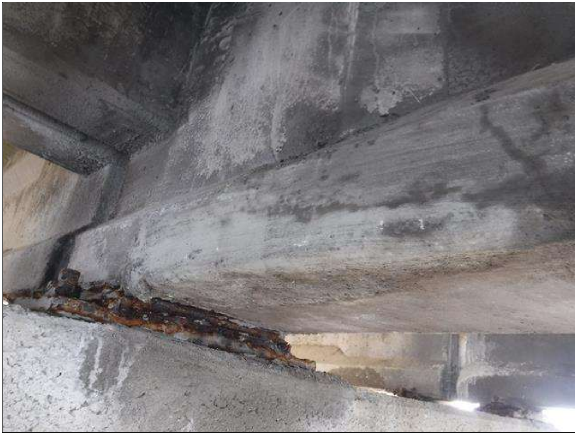
Span 160 Beam 3: 24" LONG X 7" TALL PATCHED AREA ON NORTH FACE AT BENT 160
