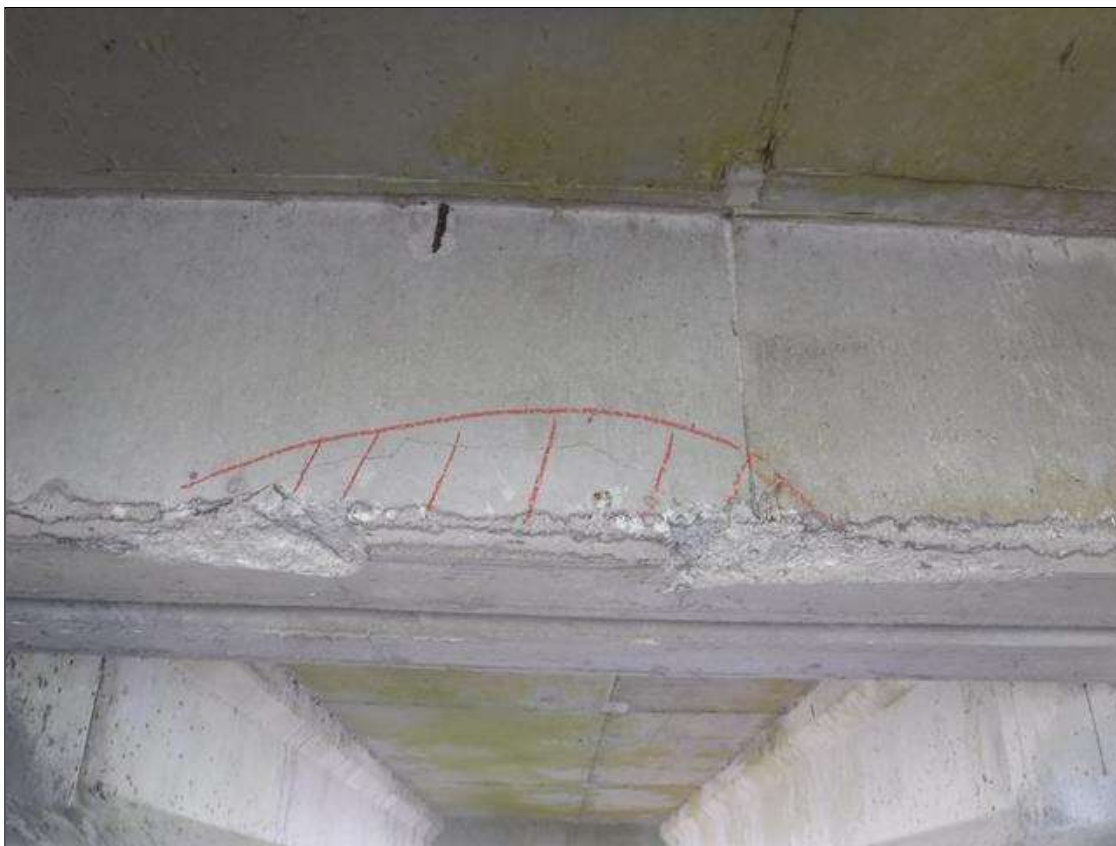
Span 129 Beam 1: 4' X 1' X 4" DEEP SPALL WITH SURROUNDING DELAMINATION, EAST FACE OF BENT 128 DIAPHRAGM, BETWEEN BEAMS 1 AND 2
