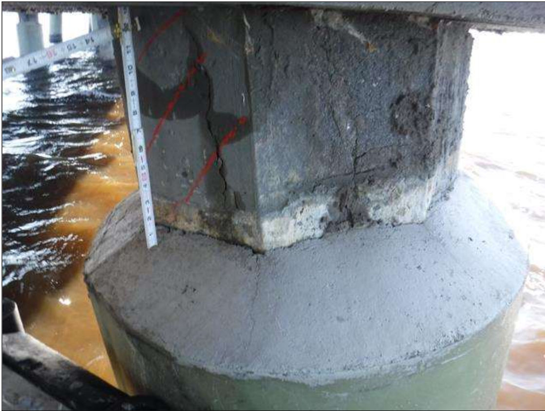
Bent 9 Saved Pile 6: PILE REPAIRED WITH 3' DIAMETER CONCRETE JACKET STARTING 12" BELOW BOTTOM OF CAP, WITH 12" X 12" AREA OF DELAMINATION ON WEST FACE
