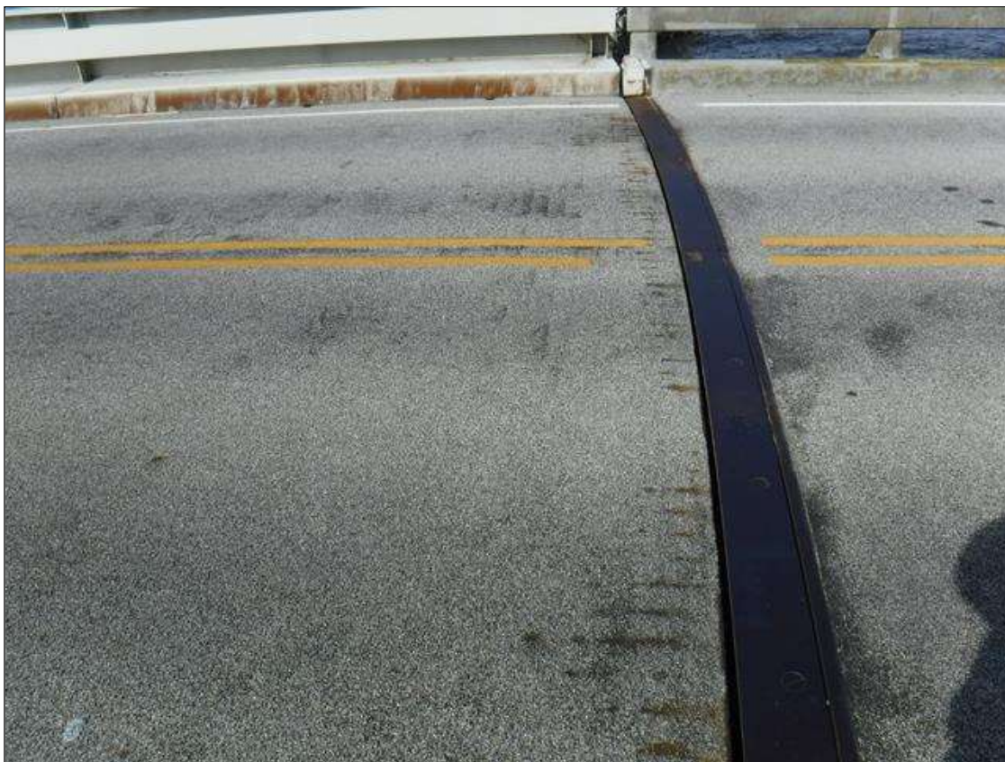
EXPANSION JOINT OVER BENT 10
