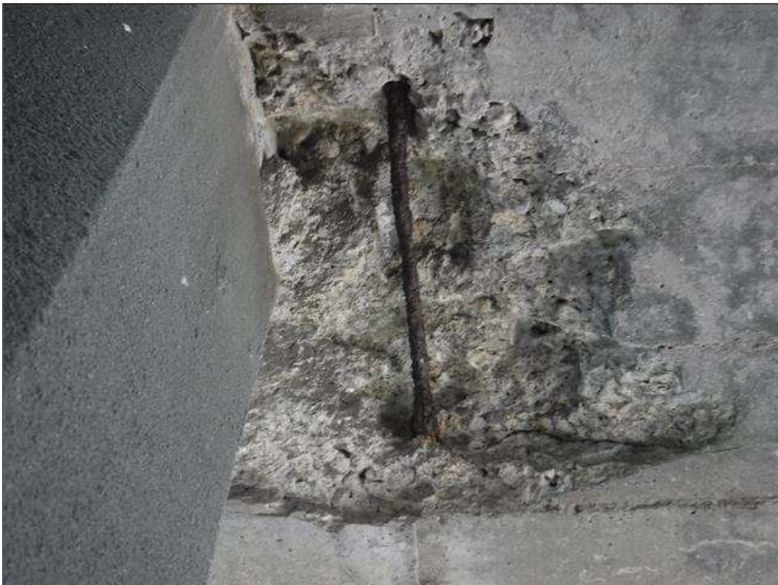
Bent 23 Cap 1: (PAR) 12" LONG, 12" TALL, AND 6" DEEP SPALL WITH EXPOSED REBAR IN BOTTOM OF BENT 23 CAP AT PILE 2. REBAR HAS 10% SECTION LOSS
