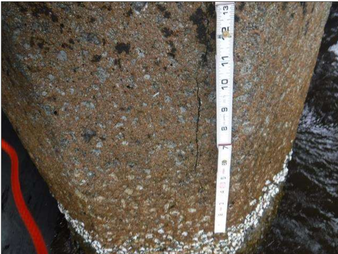
Bent 191 Pile 4: (PAR) HAIRLINE TO 1/8" CRACKS, 8' BELOW CAP, DOWN 4' , MULTIPLE FACES. SCALING TO 1" DEEP WITH LOOSE AGGREGATE FROM WATERLINE TO MUDLINE.
