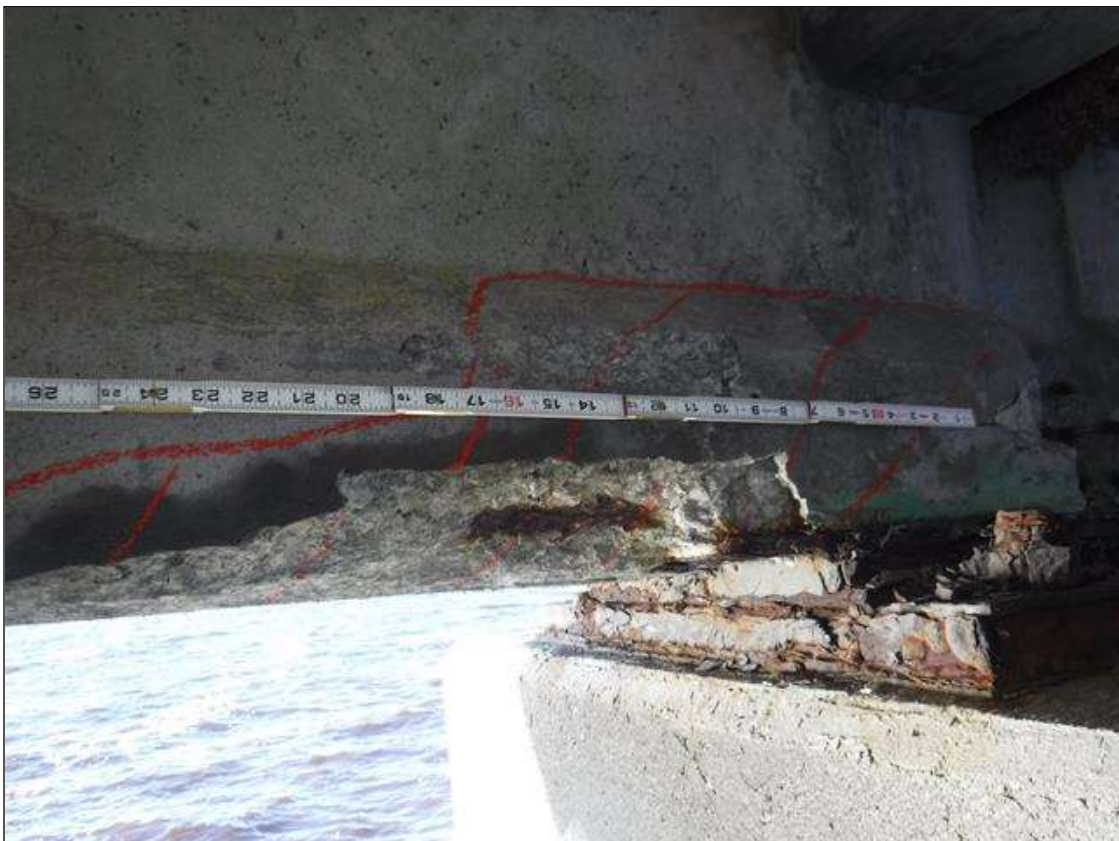
Span 10 Beam 4: (PAR) SPALL WITH EXPOSED STRAND IN GIRDER IN BOTTOM BULB OVER BENT 9 BEARING. AREA IS 10" TALL, 34" LONG, AND 6" DEEP.
