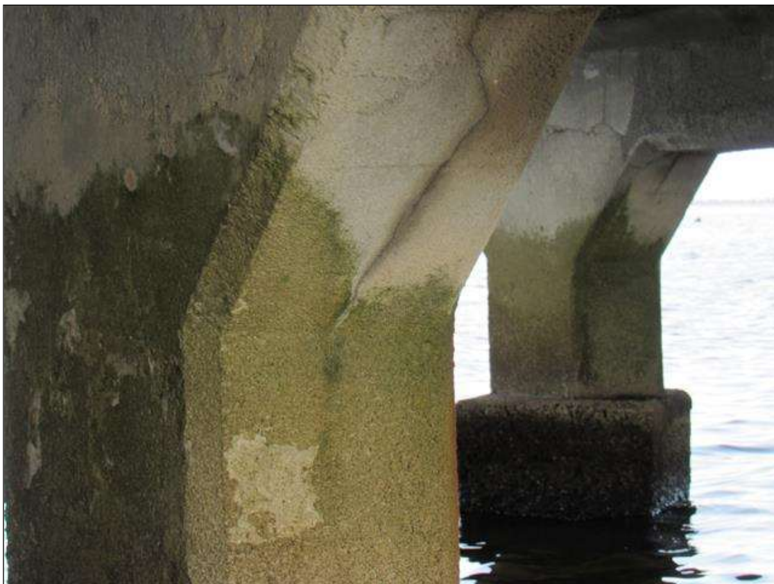
Bent 278 Pile 3: 18" X HAIRLINE VERTICAL CRACKS, WITH RUST STAINING, AT RANDOM THROUGHOUT.
