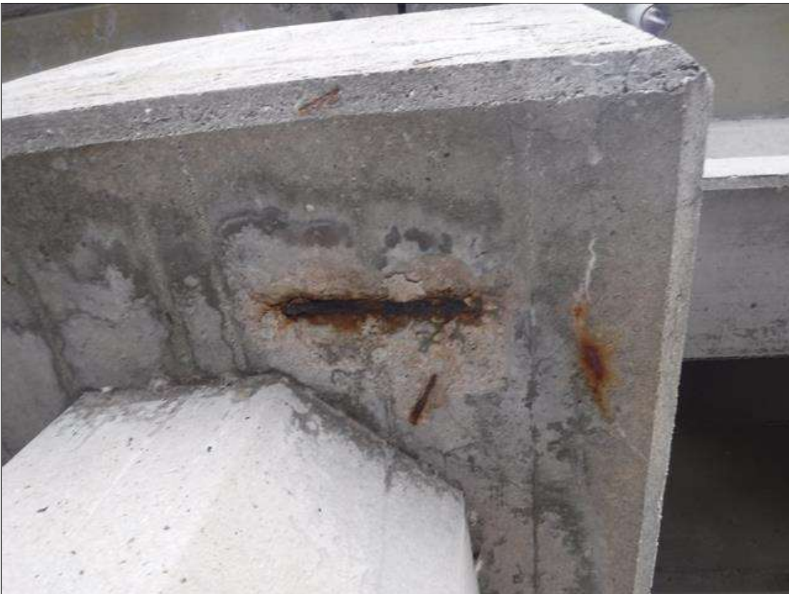
Bent 255 Cap 1: (PAR) 4" LONG, 9" WIDE AND 1" DEEP SPALL WITH EXPOSED REBAR IN BOTTOM OF RIGHT OVERHANG.
