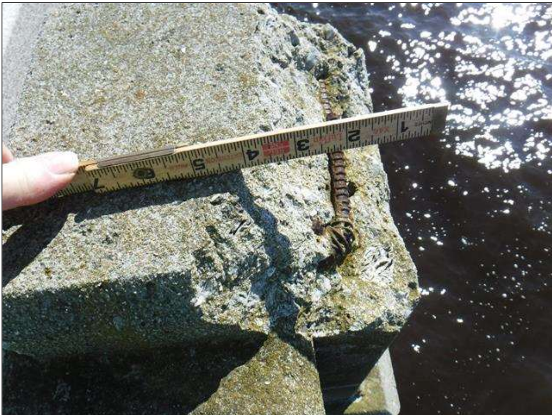
Span 25 Right Bridge Rail: 10" X 5" X 4" SPALL WITH EXPOSED REBAR ON RIGHT FACE LOCATED 5TH POST FROM BENT 24
