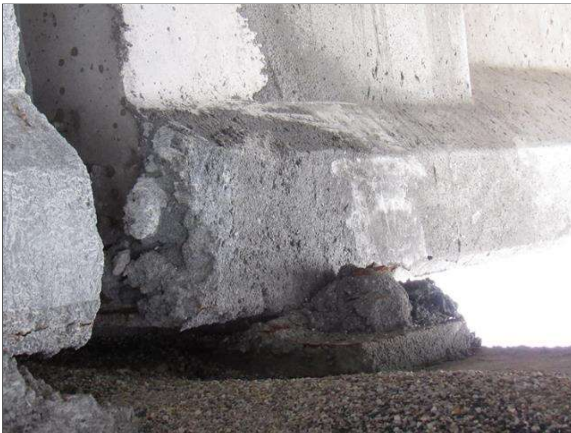
Span 47 Beam 2: 9" X 10" PATCHED AREA, SOUTH FACE, AT BENT 46.
