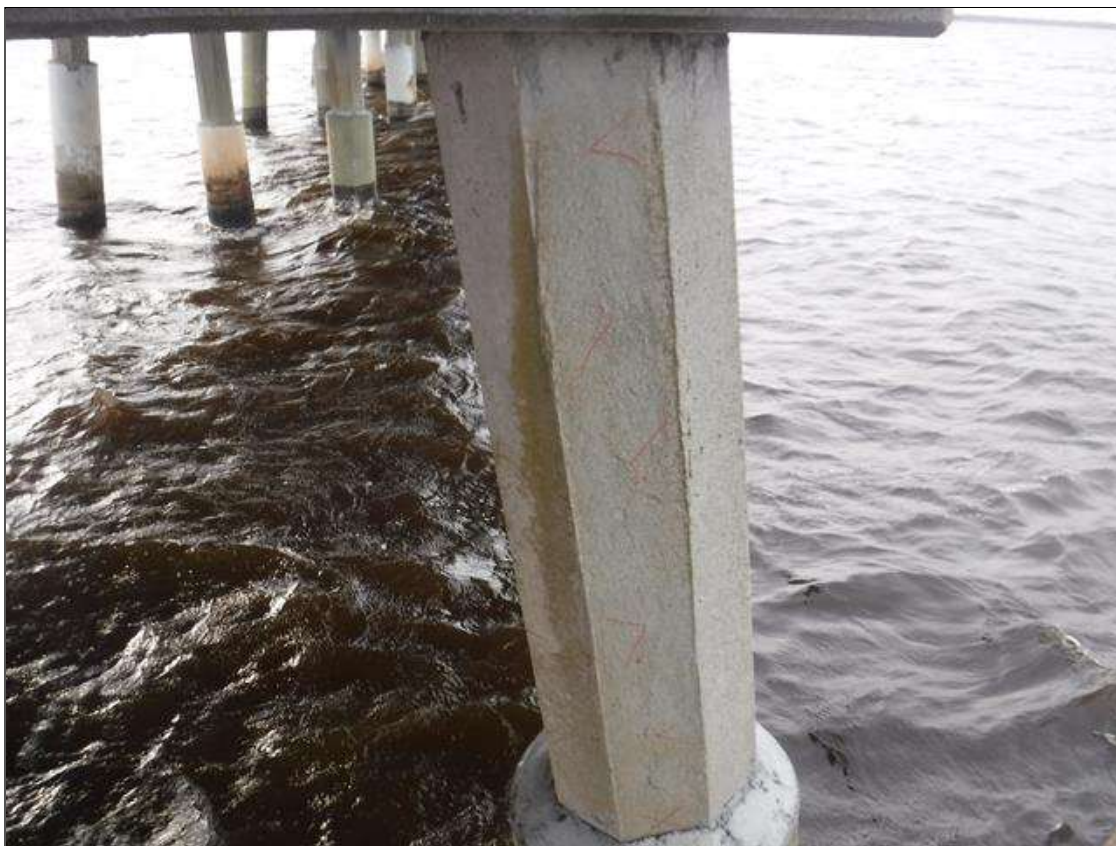
Bent 137 Pile 1: (PAR) 6' X UP TO 0.031" VERTICAL CRACK ON EAST FACE, BEGINNING AT BOTTOM OF CAP.
