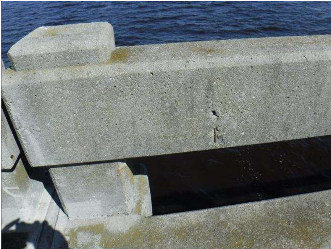
Span 49 Left Bridge Rail: 5" X 1" X 1/2" SPALL WITH EXPOSED REBAR ON RIGHT FACE LOCATED 2' FROM BENT 48
