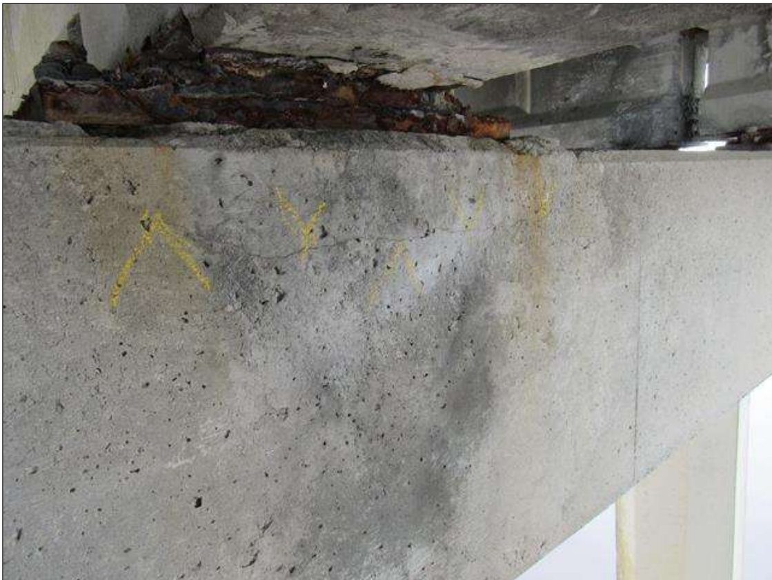
Bent 31 Cap 1: 30" LONG X 1/32" WIDE HORIZONTAL CRACK ON EAST FACE LOCATED BELOW BEAM 2
