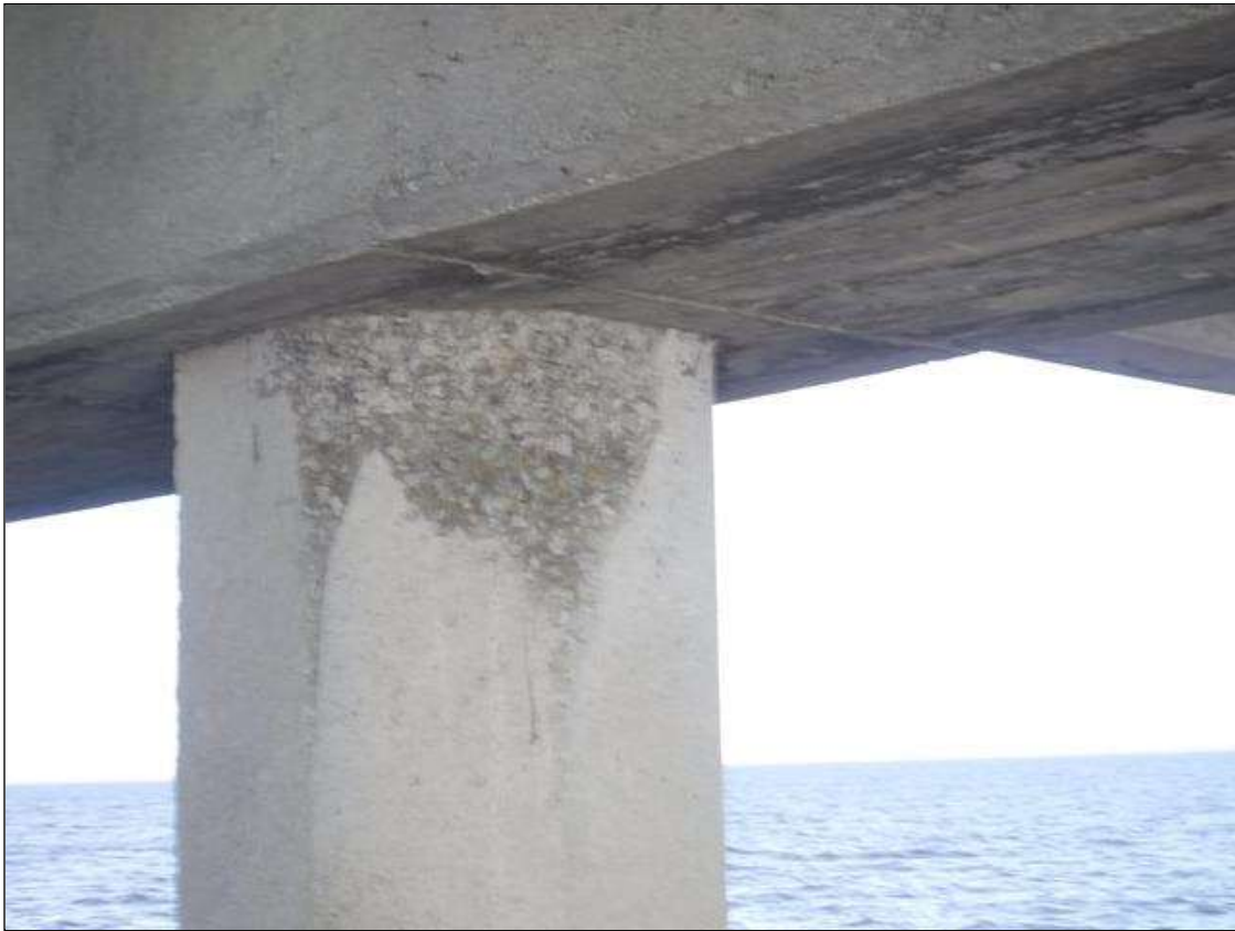
Bent 122 Pile 2: 12" X 16" X 1" SPALL, SOUTH FACE, AT BOTTOM OF CAP.
