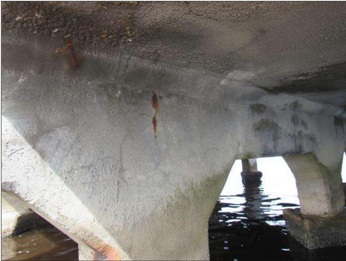
Bent 281 Cap 1: 6" HAIRLINE VERTICAL CRACK, WITH RUST STAINING, EAST FACE, ABOVE PILE 4.
