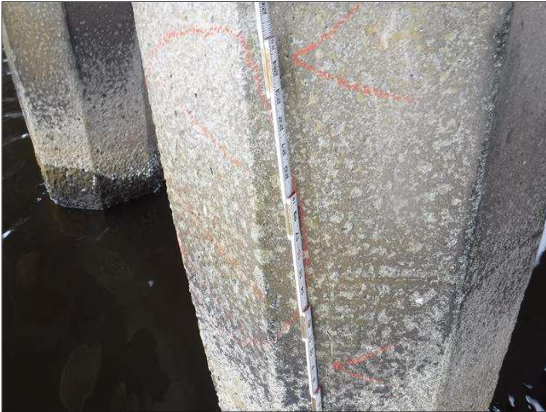
Bent 243 Pile 2: (PAR) (2) UP TO 3' X 0.03" VERTICAL CRACKS WITH SURROUNDING DELAMINATION ON NORTH FACE, BEGINNING 7' FROM BOTTOM OF CAP.
