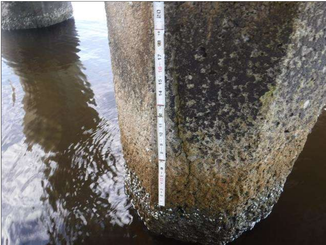
Bent 204 Pile 3: (PAR) HAIRLINE TO 1/8" CRACKS, 8' BELOW CAP, DOWN 4', MULTIPLE FACES. SCALING TO 1" DEEP WITH LOOSE AGGREGATE FROM WATERLINE TO MUDLINE.
