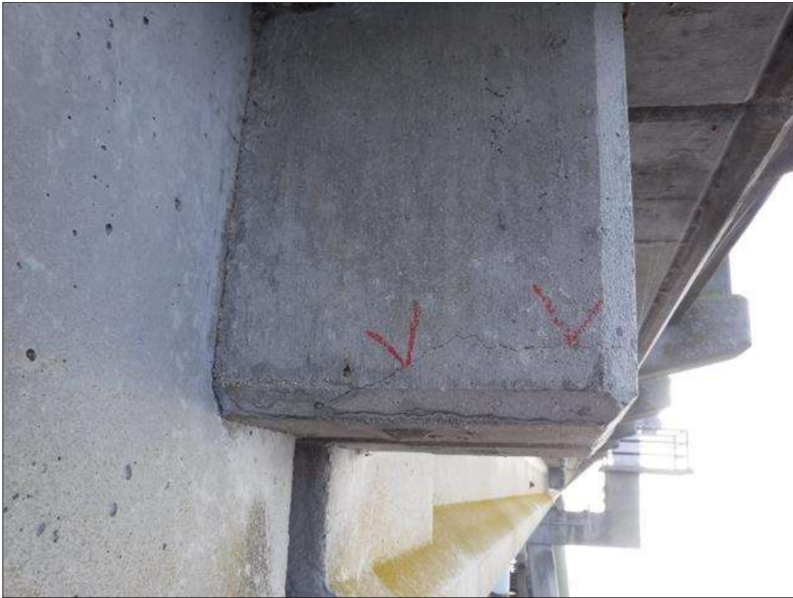
Span 121 Beam 4: 1' HAIRLINE CRACK WITH 6" SURROUNDING DELAMINATION IN WEST FACE OF SOUTH END DIAPHRAGM AT BENT 121
