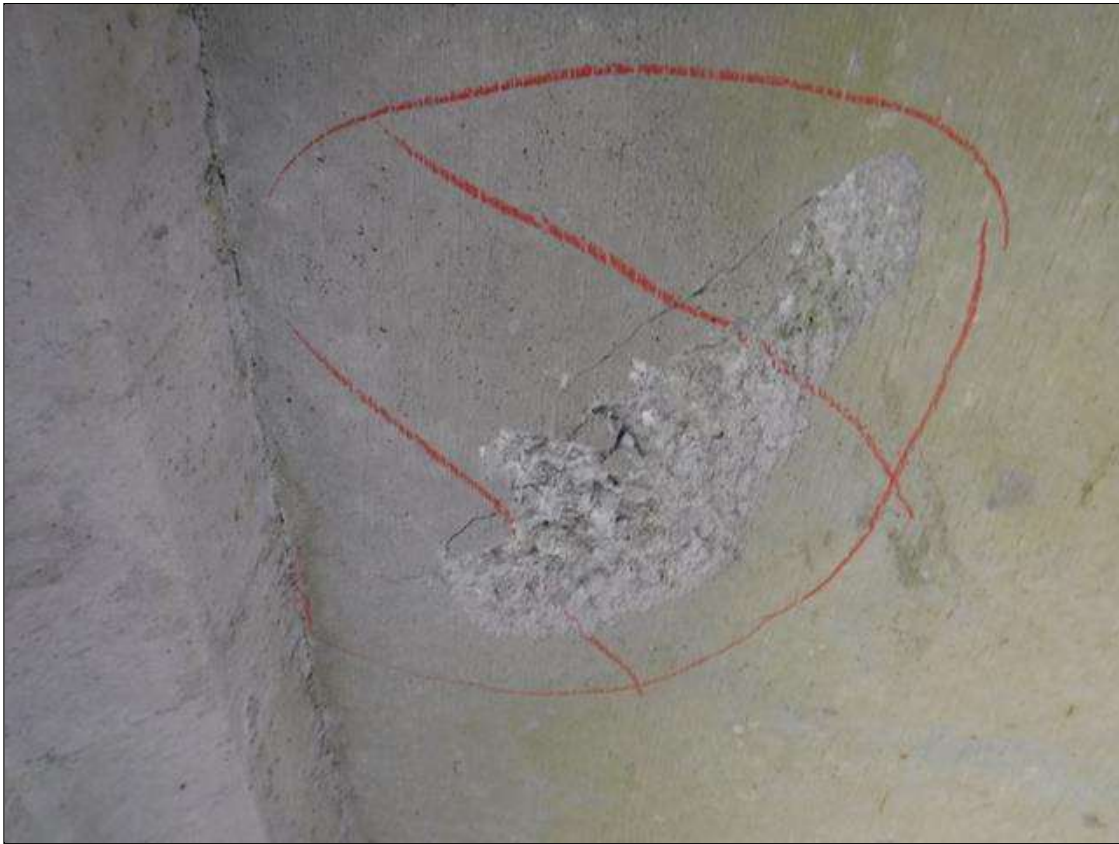
Span 228 Deck: 18" DIAMETER X 3/4" SPALL, DECK UNDERSIDE, BETWEEN BEAMS 3 AND 4, 6' FROM BENT 227, WITH ADJACENT 1' X 1' DELAMINATION.
