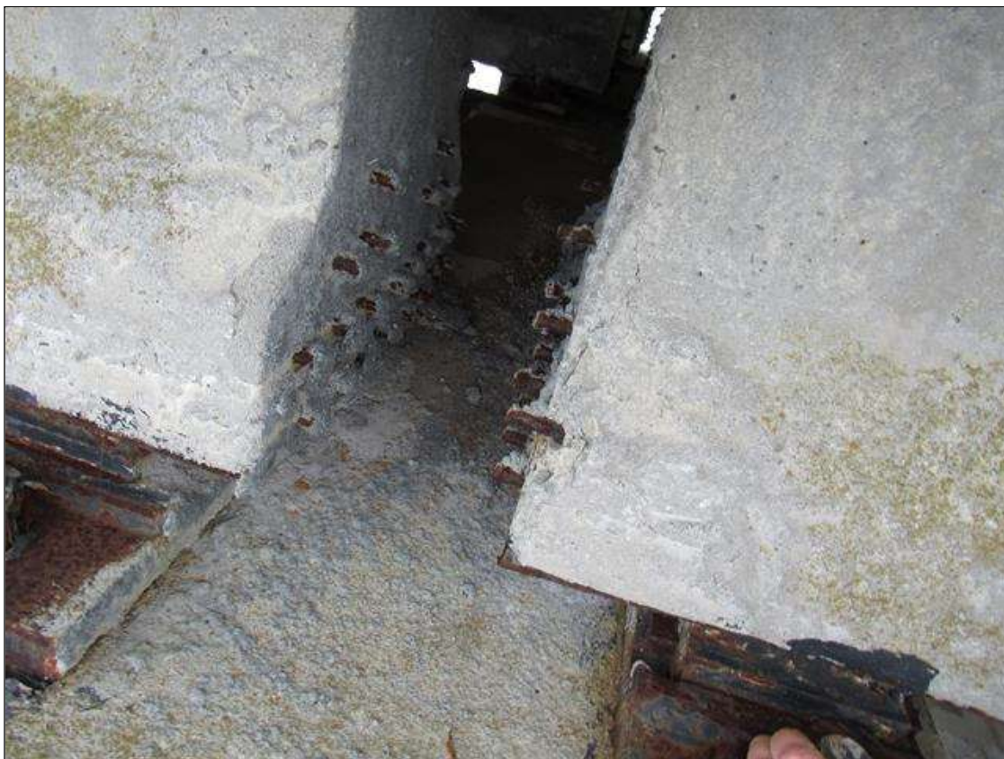
Span 69 Beam 1: 2" X 6" HIGH X 2" CORNER SPALL, NORTH FACE, AT BENT 69.
