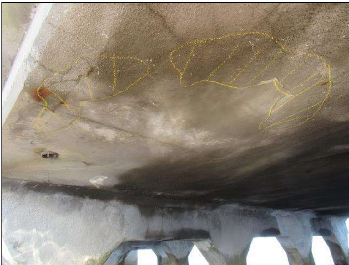
Span 281 Deck: 44" X 42" DELAMINATION ON BOTTOM FACE LOCATED RIGHT SIDE NEAR MID-SPAN
