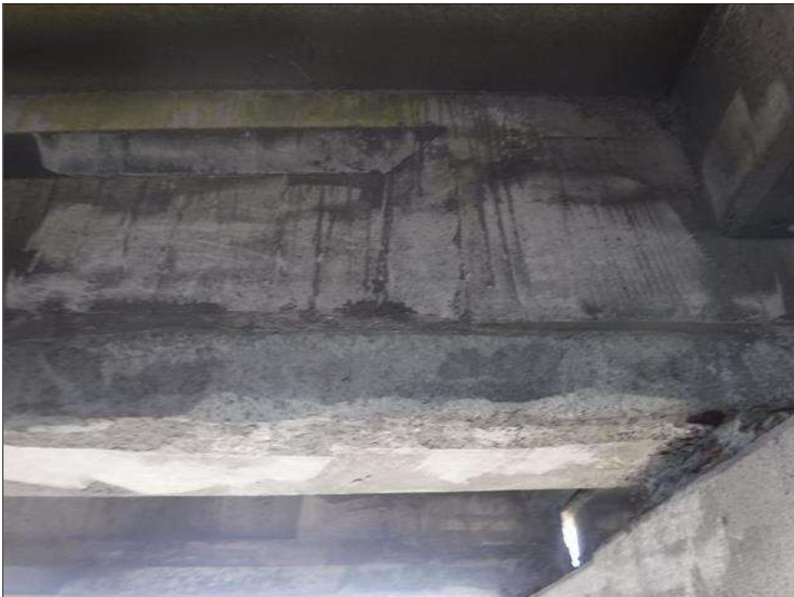
Span 27 Beam 3: 54" X 12" PATCH ON NORTH FACE AT BENT 26.
