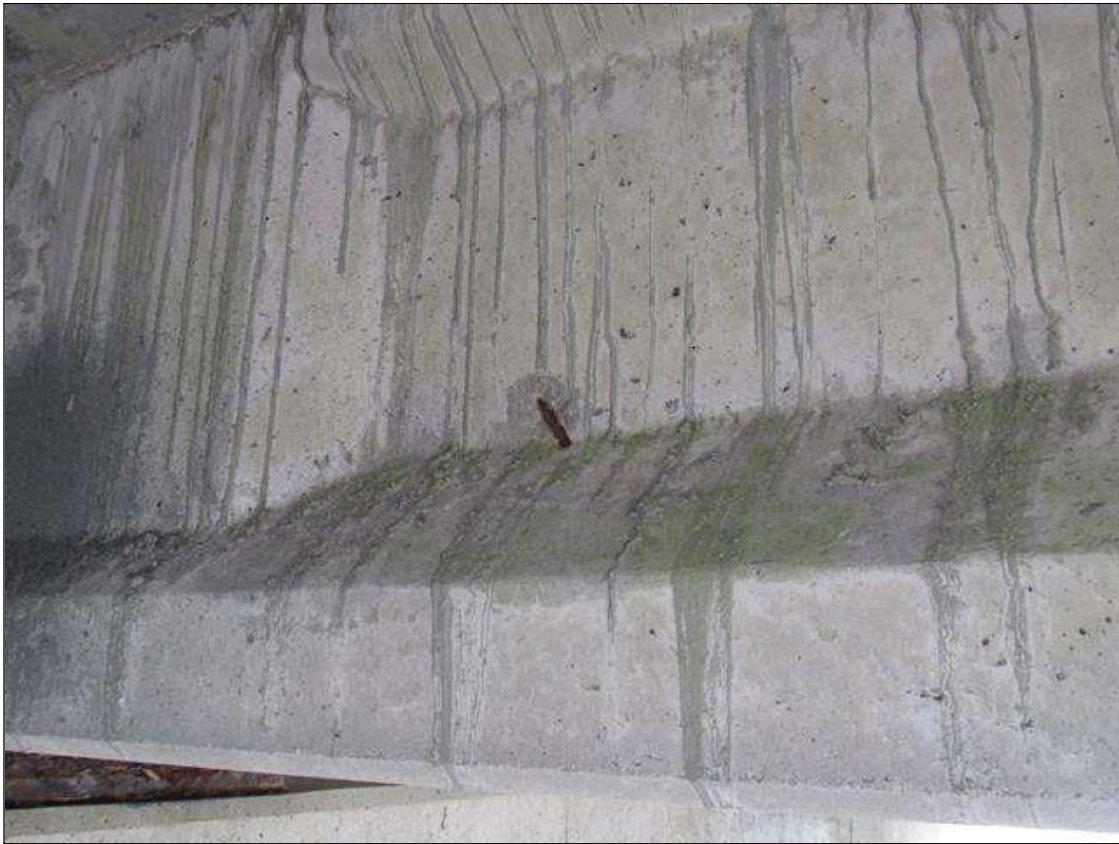
Span 67 Beam 2: 3" X 3" X 1/4" SPALL, WITH EXPOSED REBAR, NORTH FACE, 4' FROM BENT 67.
