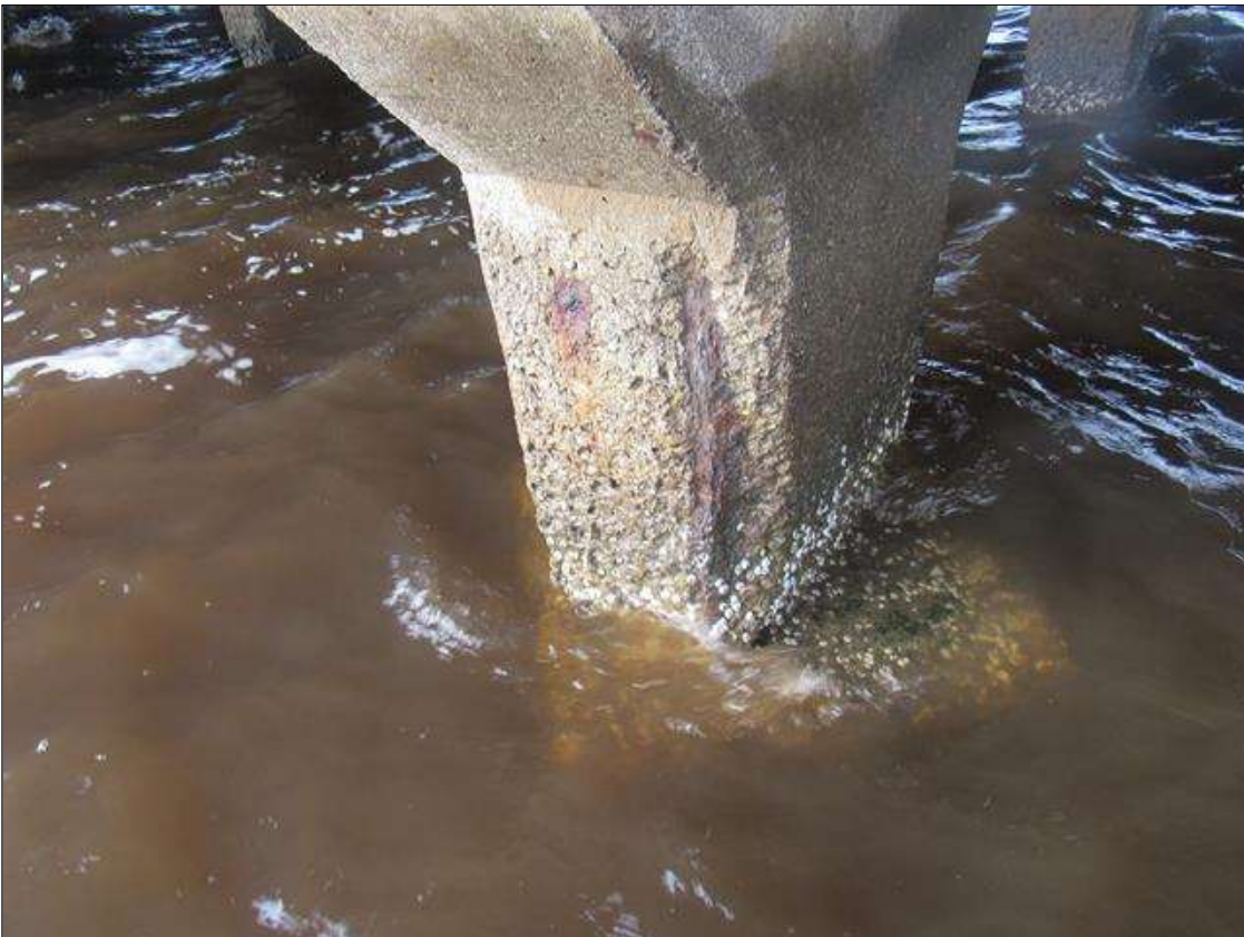
Bent 293 Pile 4: (PAR) 18" X 3" X 3" SPALL, WITH EXPOSED PRIMARY REINFORCING, SOUTHWEST CORNER, AT BOTTOM OF CAP. REBAR HAS 10% SECTION LOSS
