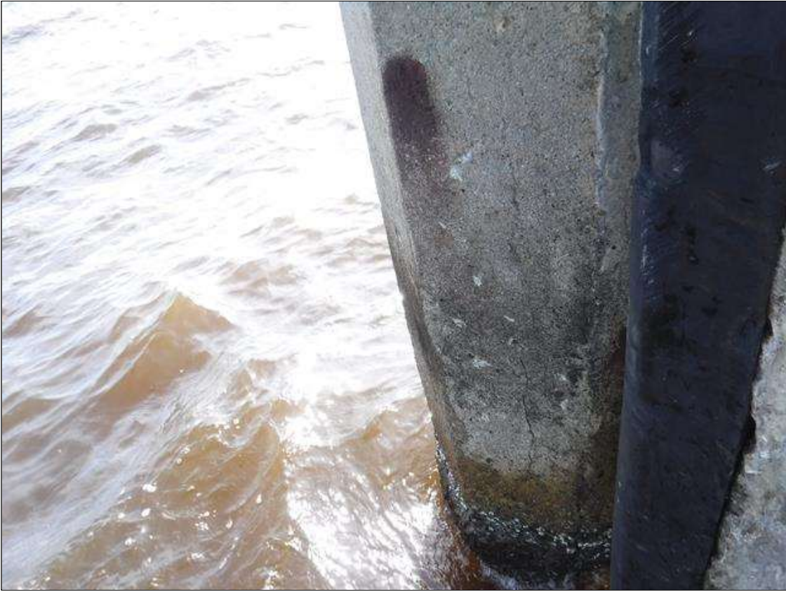
Bent 126 Pile 4: 3' X 1' DELAMINATION, EAST FACE, 8' FROM BOTTOM OF CAP, EXTENDING BELOW WATERLINE.
