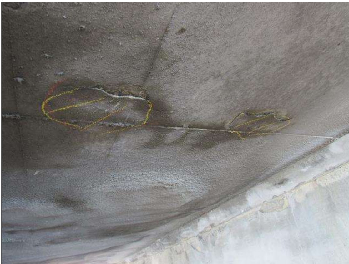
Span 278 Deck: 5 SF OF DELAMINATION ON DECK UNDERSIDE, AT RANDOM THROUGHOUT
