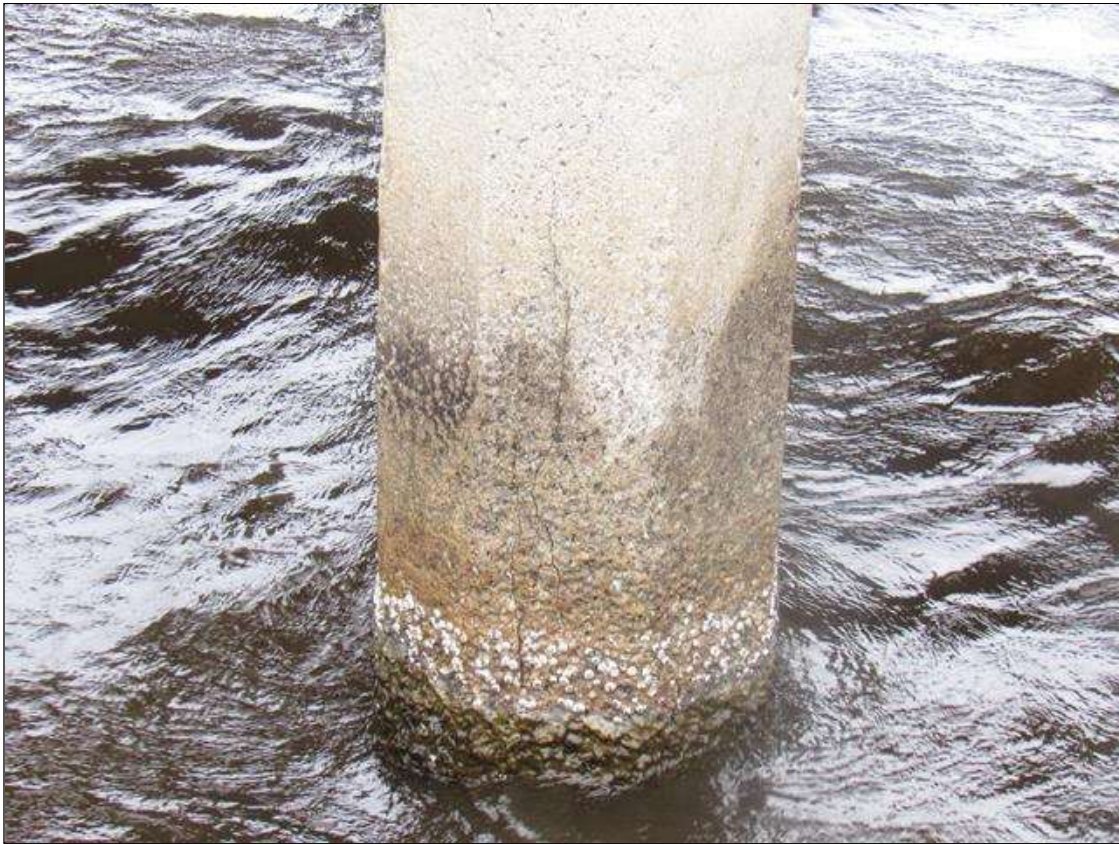
Bent 100 Pile 4: 2' X UP TO 0.007" VERTICAL CRACKS, WEST FACE, BEGINNING 9' FROM BOTTOM OF CAP, WITH ADJACENT 2' X UP TO 1.5' DELAMINATION.
