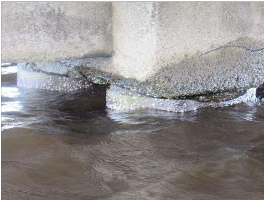
Bent 275 Cap 1: 5' X UP TO 6" X 6" SPALL, WITH EXPOSED REINFORCING, NORTH FACE OF PILE 2 BLOCK-OUT.
