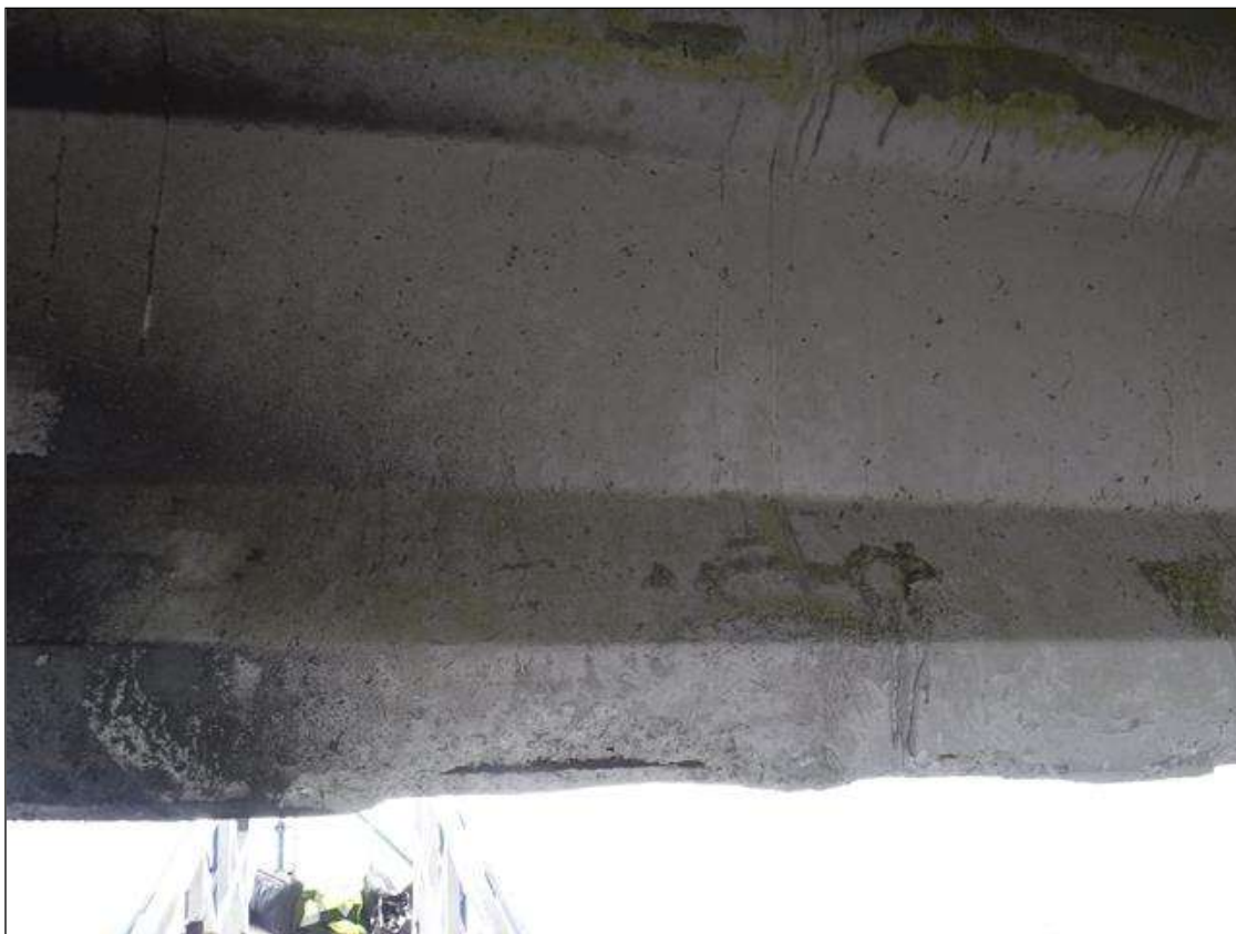
Span 97 Beam 3: (PAR) (3) UP TO 18" LONG X 5" WIDE X 6" SPALL WITH EXPOSED STRANDS ON NORTH FACE 25' FROM BENT 97
