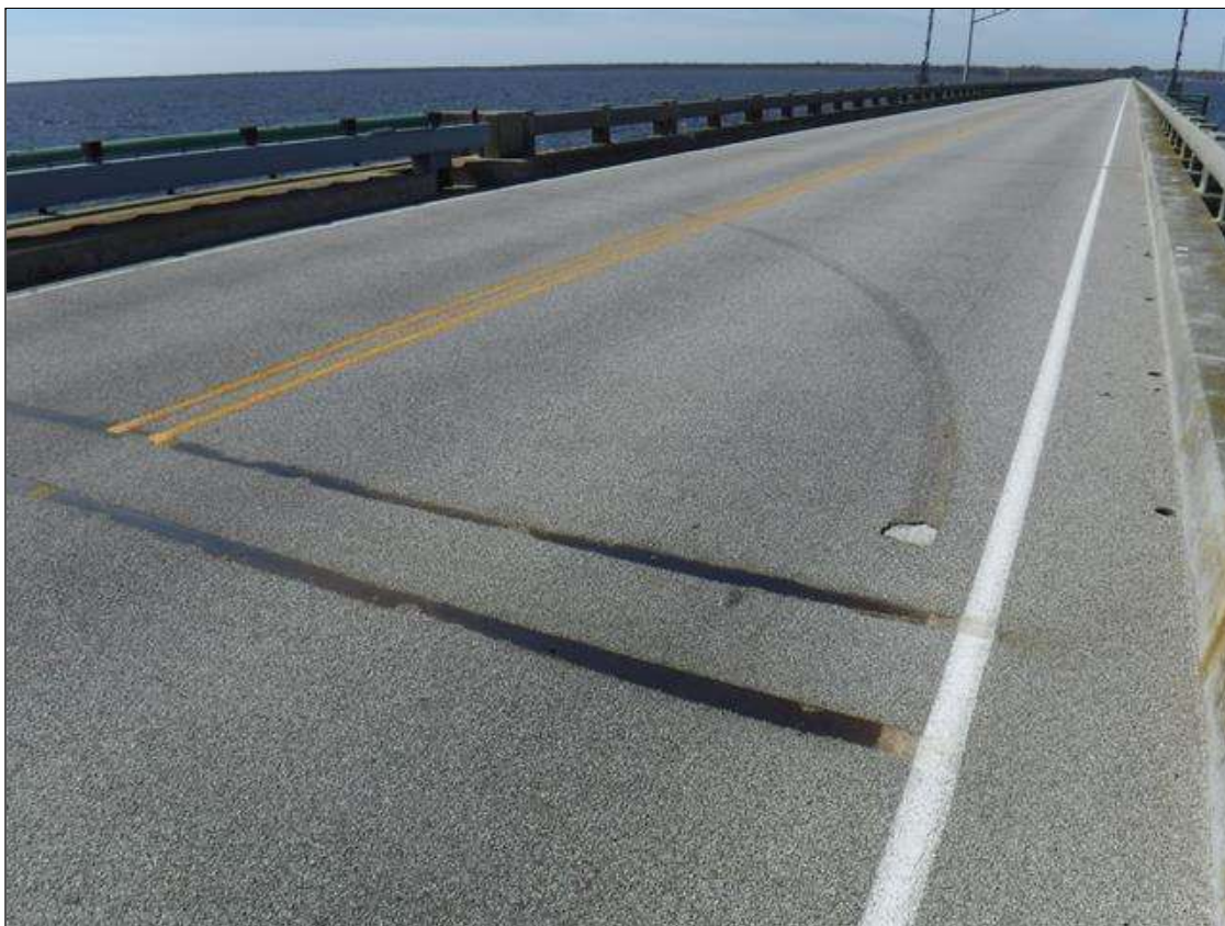
Span 113 Wearing Surface: (PAR) 10" DIAMETER SPALL IN LEFT TRAVEL LANE, 2' FROM BENT 113 AND 2' FROM LEFT CURB
