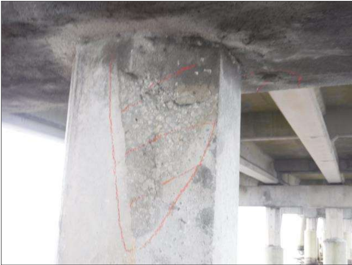
Bent 185 Pile 2: 24" X 12" X 2" SPALL, EAST FACE, BEGINNING FROM BOTTOM OF CAP.
