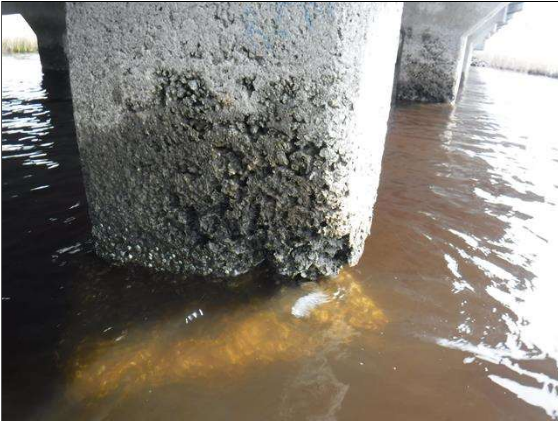
Bent 296 Pile 4: (PAR) 12" X 10" X 10" SPALL, WITH EXPOSED REBAR, SOUTHWEST CORNER, 2' FROM BOTTOM OF CAP. REBAR HAS UP TO COMPLETE SECTION LOSS
