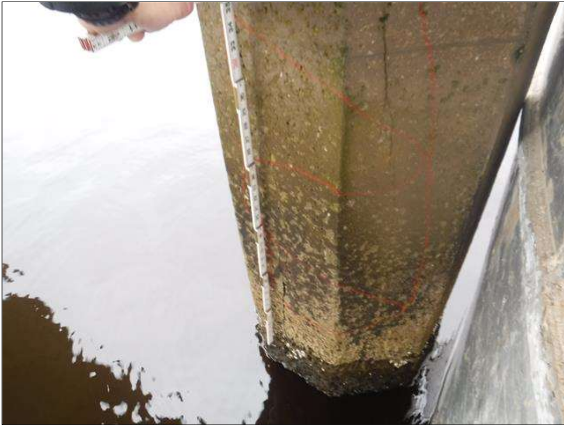
Bent 243 Pile 6: (PAR) HAIRLINE TO 1/16" CRACKS, 8' BELOW CAP, DOWN 4', NORTH FACE. SCALING TO 1" DEEP WITH LOOSE AGGREGATE FROM WATERLINE TO MUDLINE.
