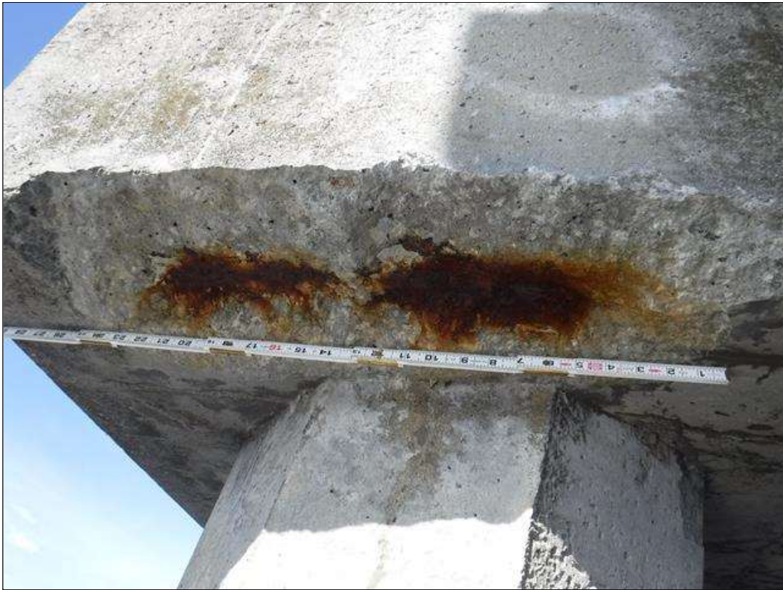
Bent 218 Cap 1: (PAR) 2.5' X UP TO 10" X 2.5" SPALL, WITH EXPOSED REBAR, EAST FACE, AT PILE 4. REBAR HAS 10% SECTION LOSS.
