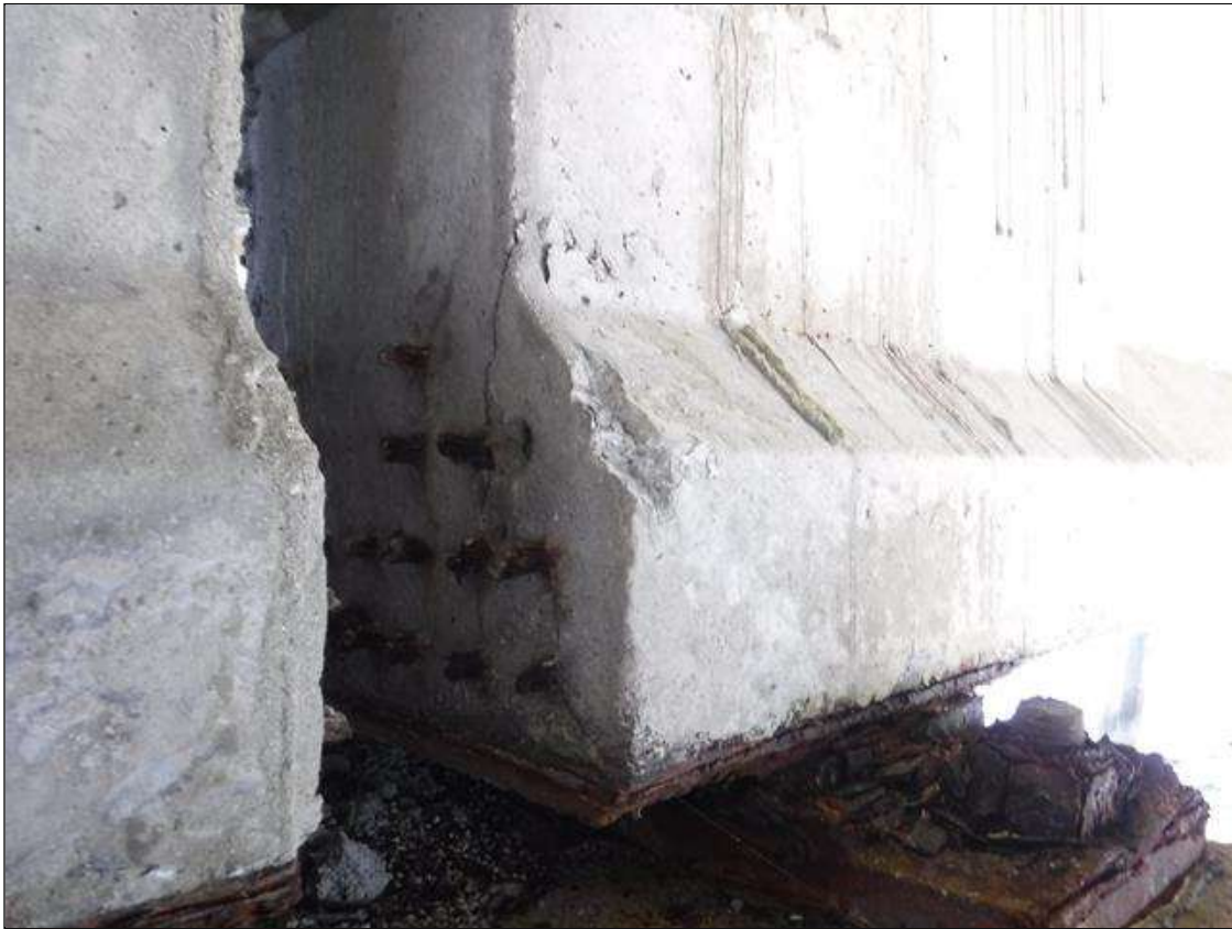
Span 146 Beam 3: 6" X 6" DELAMINATION ON SOUTH FACE AT BENT 146
