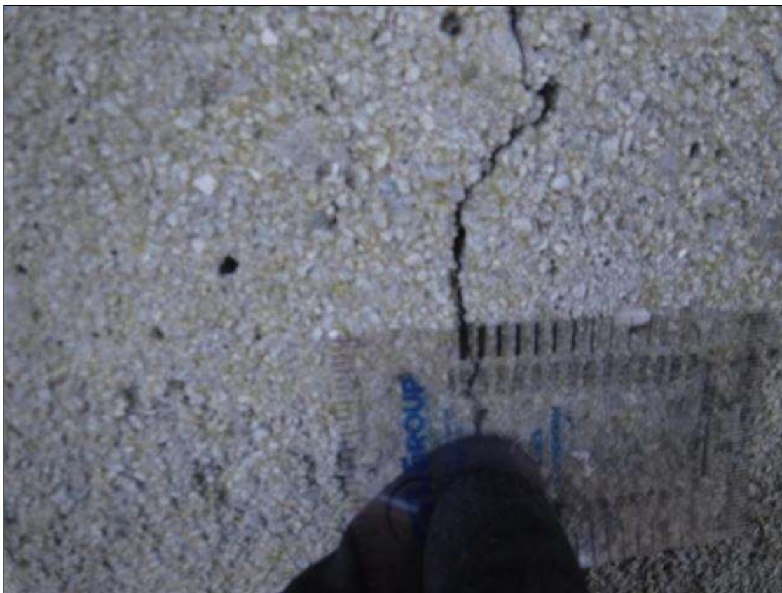
Bent 123 Pile 4: (PAR) UP TO 7' X 0.06" VERTICAL CRACKS, NORTH FACE, BEGINNING 3' FROM BOTTOM OF CAP.
