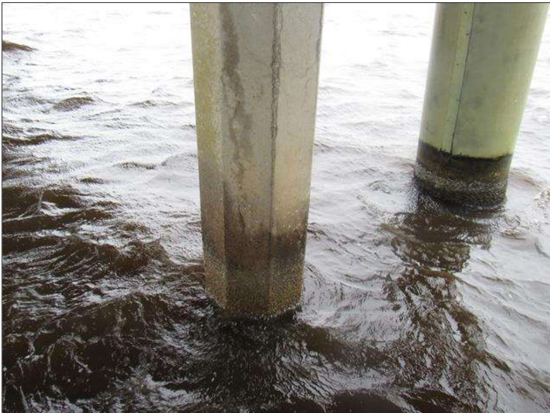
Bent 100 Pile 2: (PAR) 3' X UP TO 0.012" VERTICAL CRACKS, EAST FACE, BEGINNING 9' FROM BOTTOM OF CAP, WITH ADJACENT 3' X UP TO 2' DELAMINATION.
