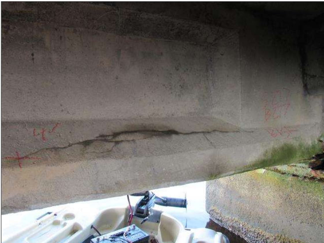
Span 277 Beam 1: (PAR) 4' LONG X 1/16" WIDE HORIZONTAL CRACKS WITH SURROUNDING DELAMINATION ON SOUTH FACE, 4' FROM BENT 277.
