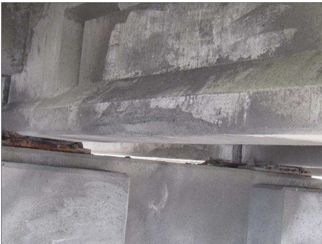
Span 45 Beam 2: 3.5' X UP TO 6" PATCHED AREA, BOTTOM FACE, EXTENDING 5" ONTO NORTH FACE, 5' FROM BENT 45.
