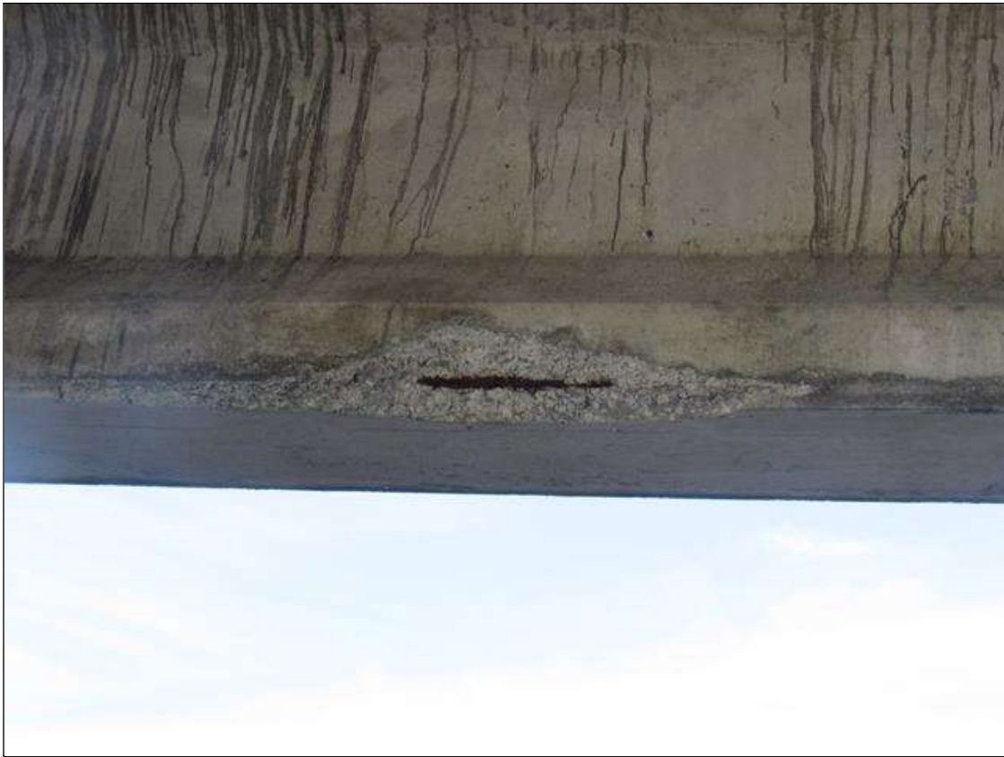
Span 8 Beam 1: (PAR) 42" X 4" X 4" EDGE SPALL WITH EXPOSED STRAND BOTTOM SOUTH CORNER, 20' FROM BENT 7.
