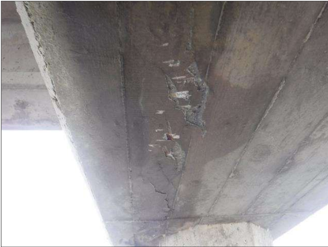
Bent 176 Cap 1: 3' X 1' DELAMINATION, BOTTOM FACE, BETWEEN BEAMS 1 AND 2
