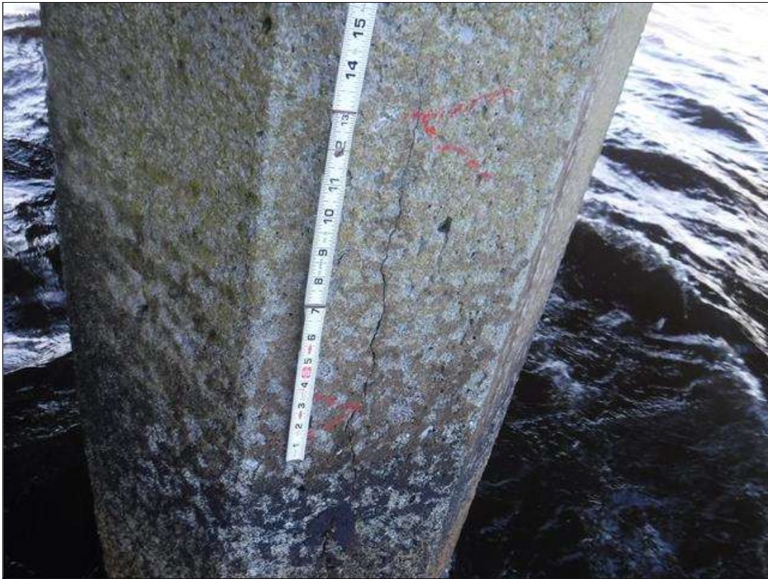
Bent 162 Pile 1: (PAR) 3' LONG X 0.06" VERTICAL CRACK ON NORTH FACE 8' BELOW CAP
