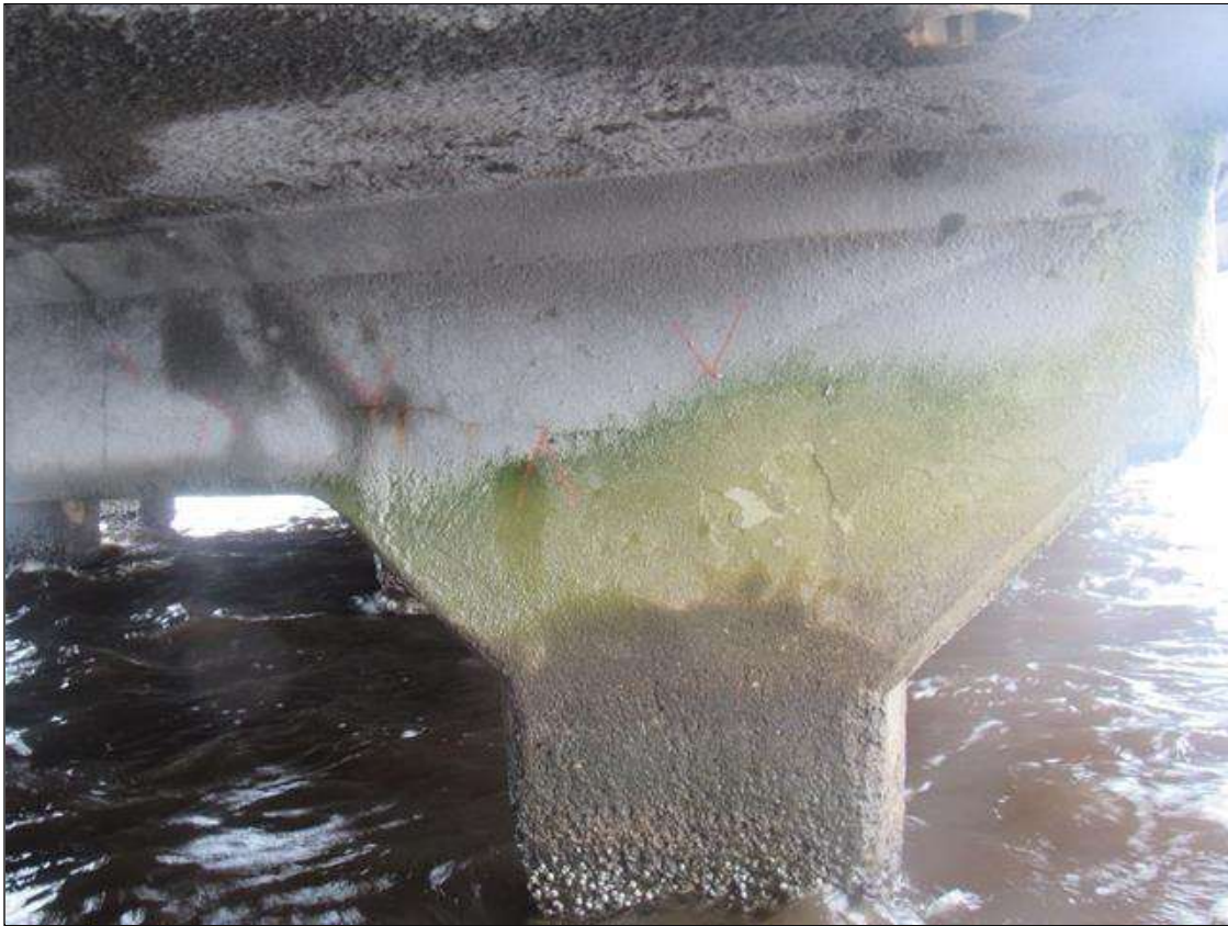
Bent 291 Cap 1: 4' OF UP TO 1/16" LONGITUDINAL CRACKS, AT RANDOM THROUGHOUT, EAST AND WEST FACES.
