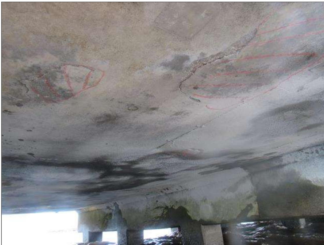
Span 295 Deck: (3) UP TO 14" X 20" DELAMINATIONS, AT NEAR RIGHT EDGE OF DECK UNDERSIDE.
