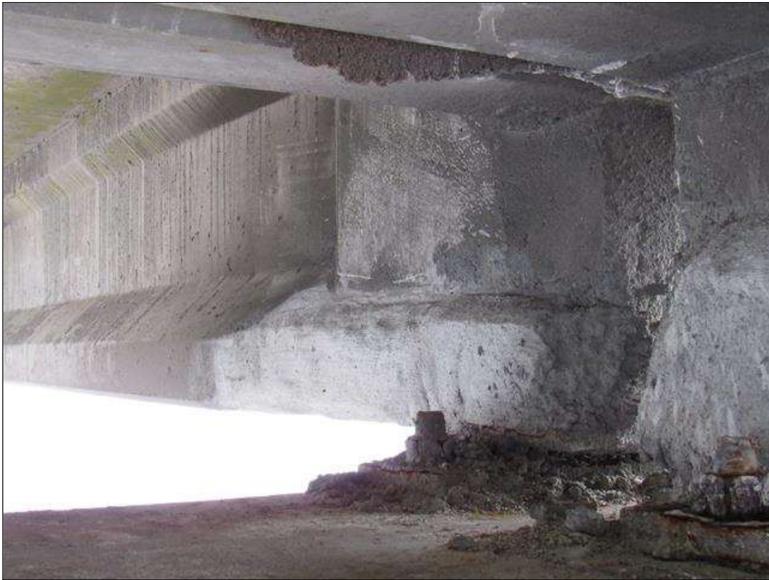
Span 60 Beam 4: 5' X 12" X 12" CORNER PATCHED AREA, NORTH FACE, AT BENT 59.
