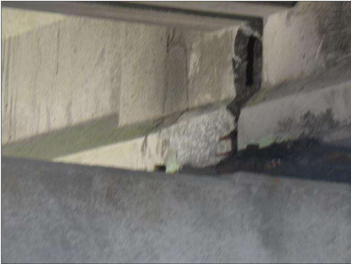
Span 7 Beam 3: (PAR) 12" X 8" X 2" SPALL WITH EXPOSED STRAND, NORTH FACE, AT BENT 7.
