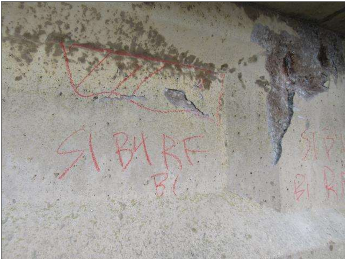
Span 1 Beam 4: 21" X 6" DELAMINATION ON RIGHT FACE LOCATED AT BENT 1
