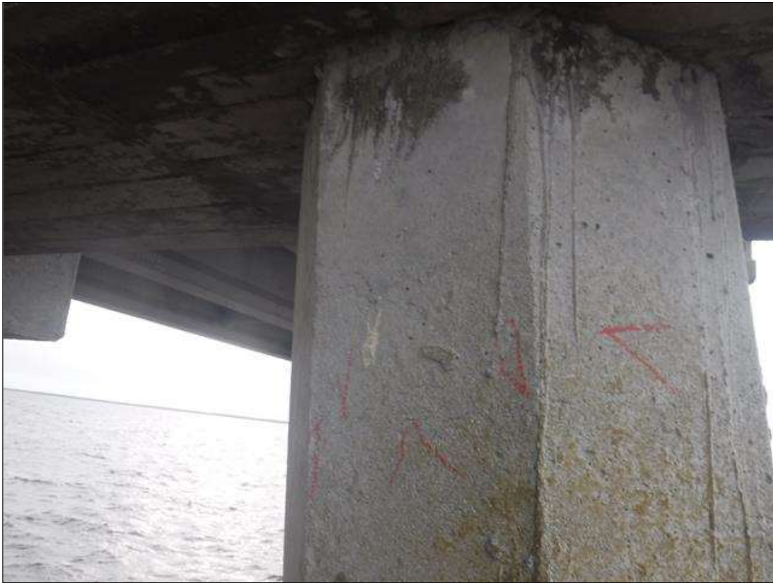
Bent 139 Pile 1: UP TO 2' X 0.009" VERTICAL CRACKS, AT RANDOM THROUGHOUT.
