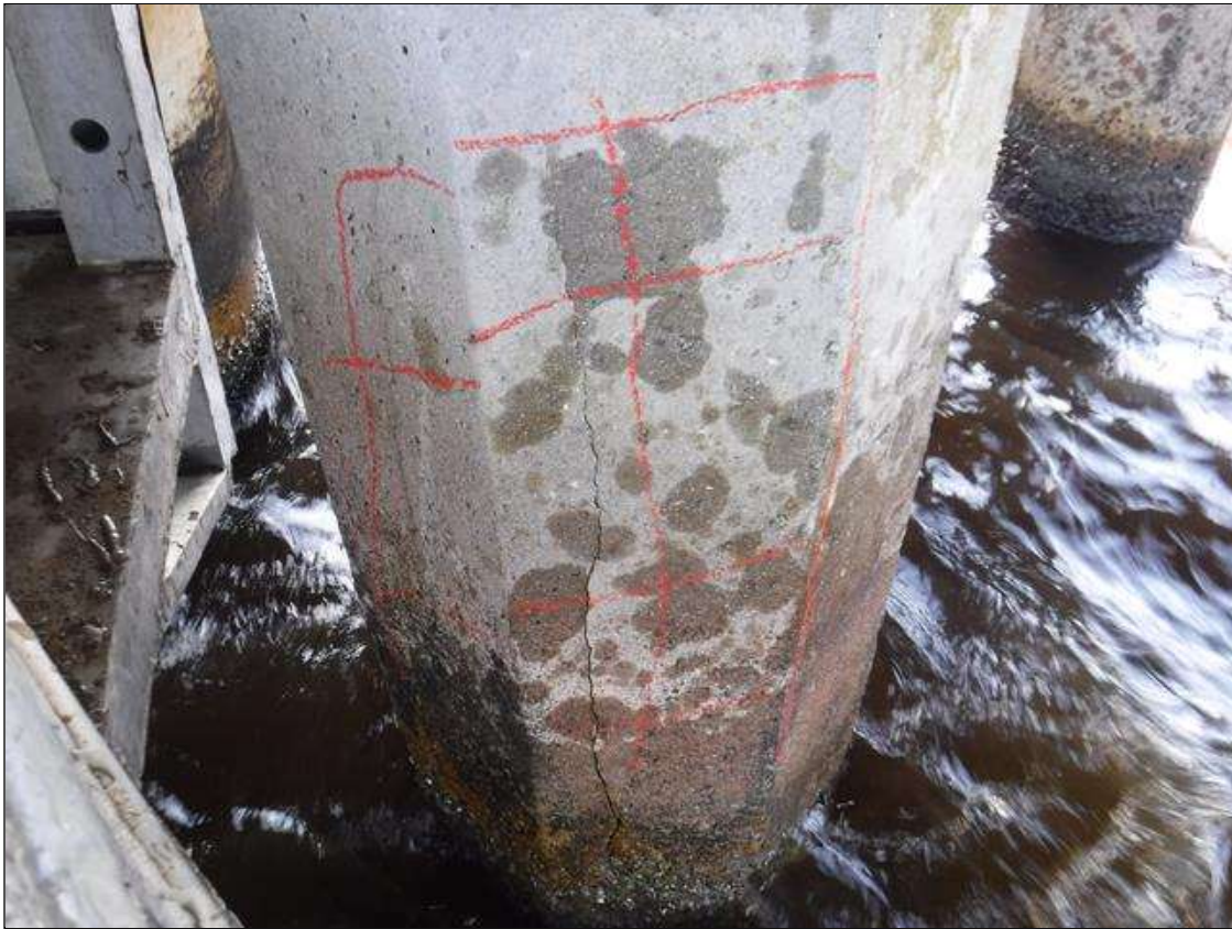
Bent 13 Saved Pile 2: 4' X 2' DELAMINATION, NORTH FACE, 5' BELOW BOTTOM OF CAP.
