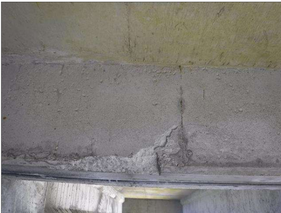
Span 147 Beam 4: 18" X 6" X 2" DEEP SPALL, WEST FACE OF BENT 147 DIAPHRAGM, BETWEEN BEAMS 3 AND 4
