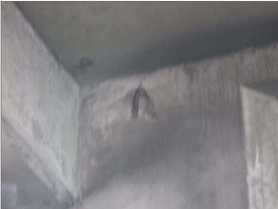
Span 13 Beam 3: 6" X 6" X 2" SPALL, WITH EXPOSED REINFORCING, TOP OF NORTH FACE, AT BENT 13.
