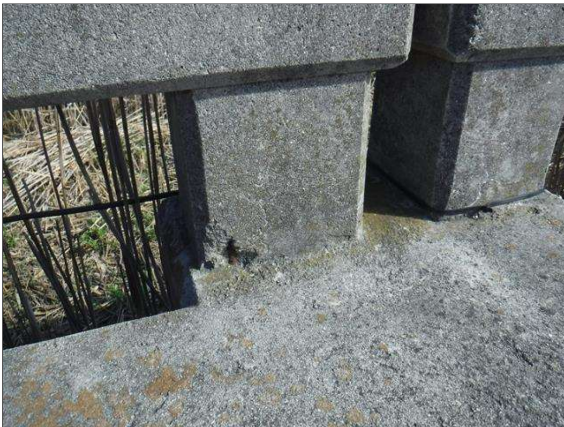
Span 312 Left Bridge Rail: 2" X 2" X 1" DEEP SPALL WITH EXPOSED REBAR AT BOTTOM RIGHT CORNER AT MID SPAN POST
