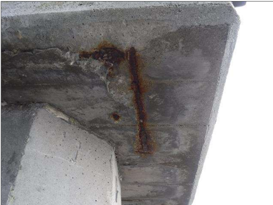
Bent 231 Cap 1: 12" X 12" X 3/4" SPALL, WITH EXPOSED REINFORCING, BOTTOM FACE, SOUTH OVERHANG.
