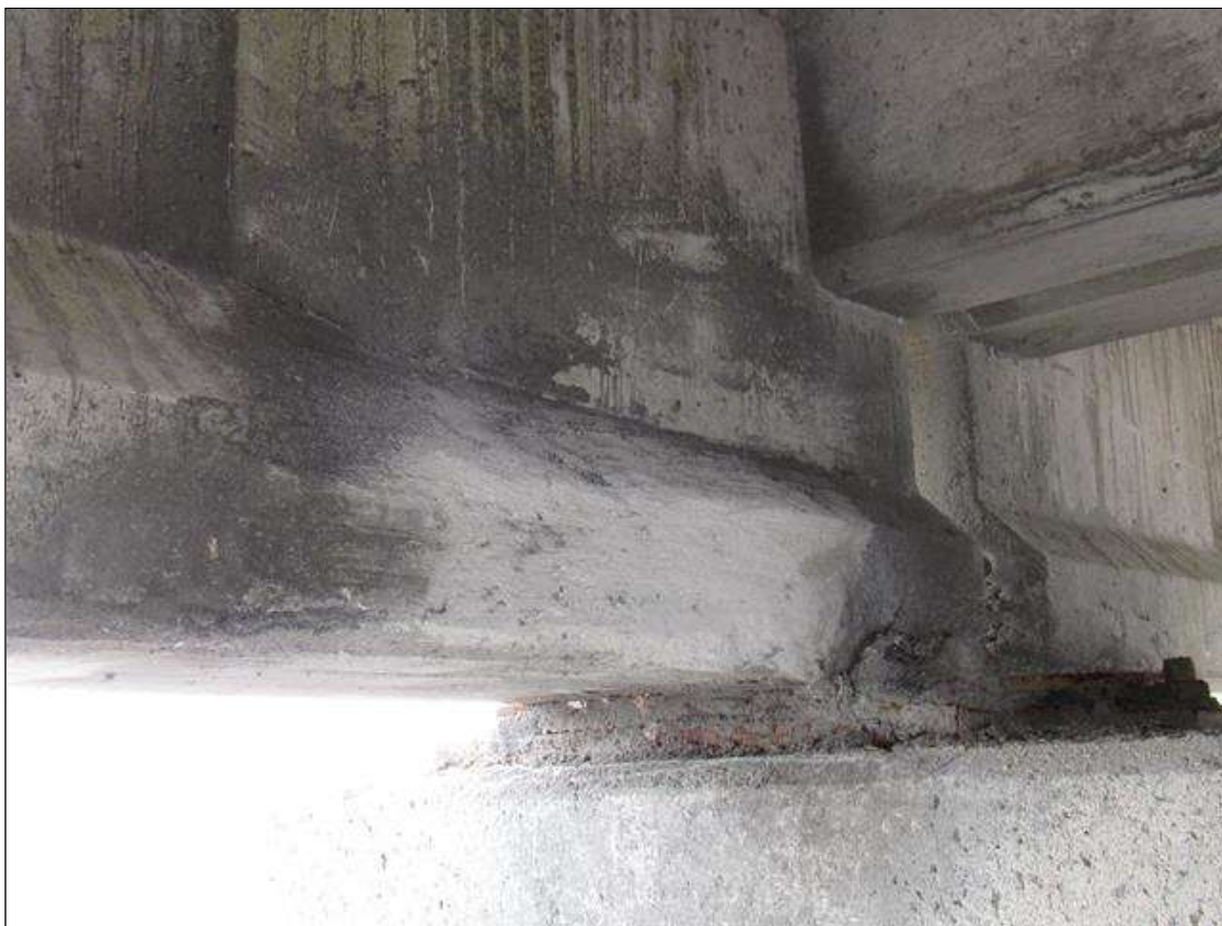
Span 62 Beam 4: 2' X 8" X 12" CORNER PATCHED AREA, NORTH FACE, AT BENT 61.
