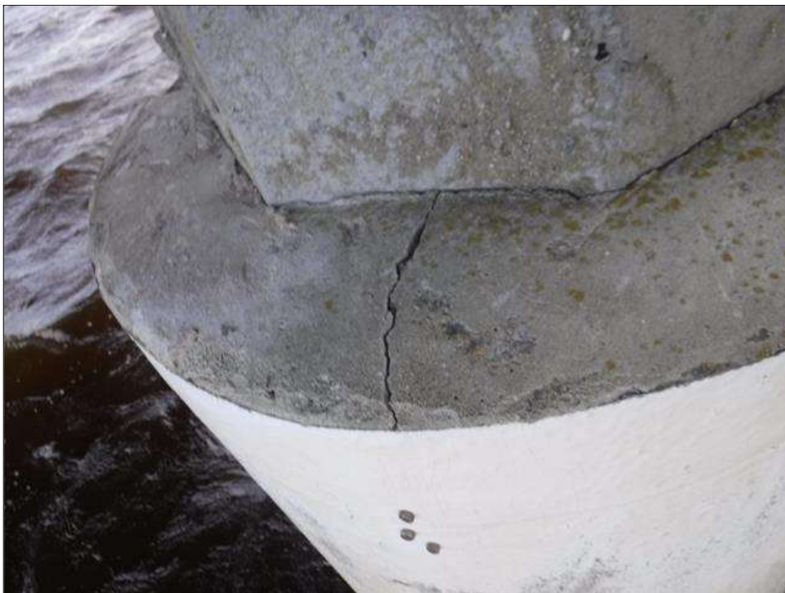
Bent 130 Pile 2: CRACKED DELAMINATION AT RANDOM THROUGHOUT, TOP OF PILE JACKET.
