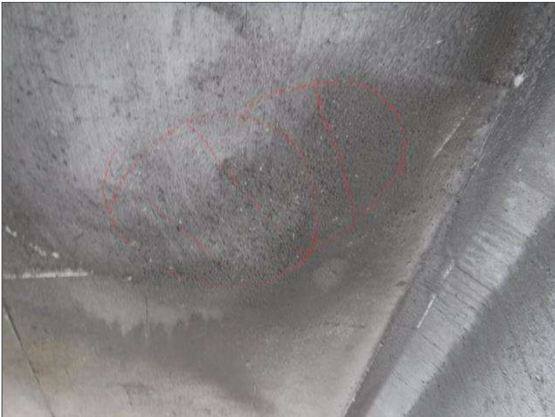
Span 233 Deck: 2' DIAMETER FAILED PATCH WITH DELAMINATION ON UNDERSIDE OF DECK IN BAY 1, 10' FROM BENT 23
