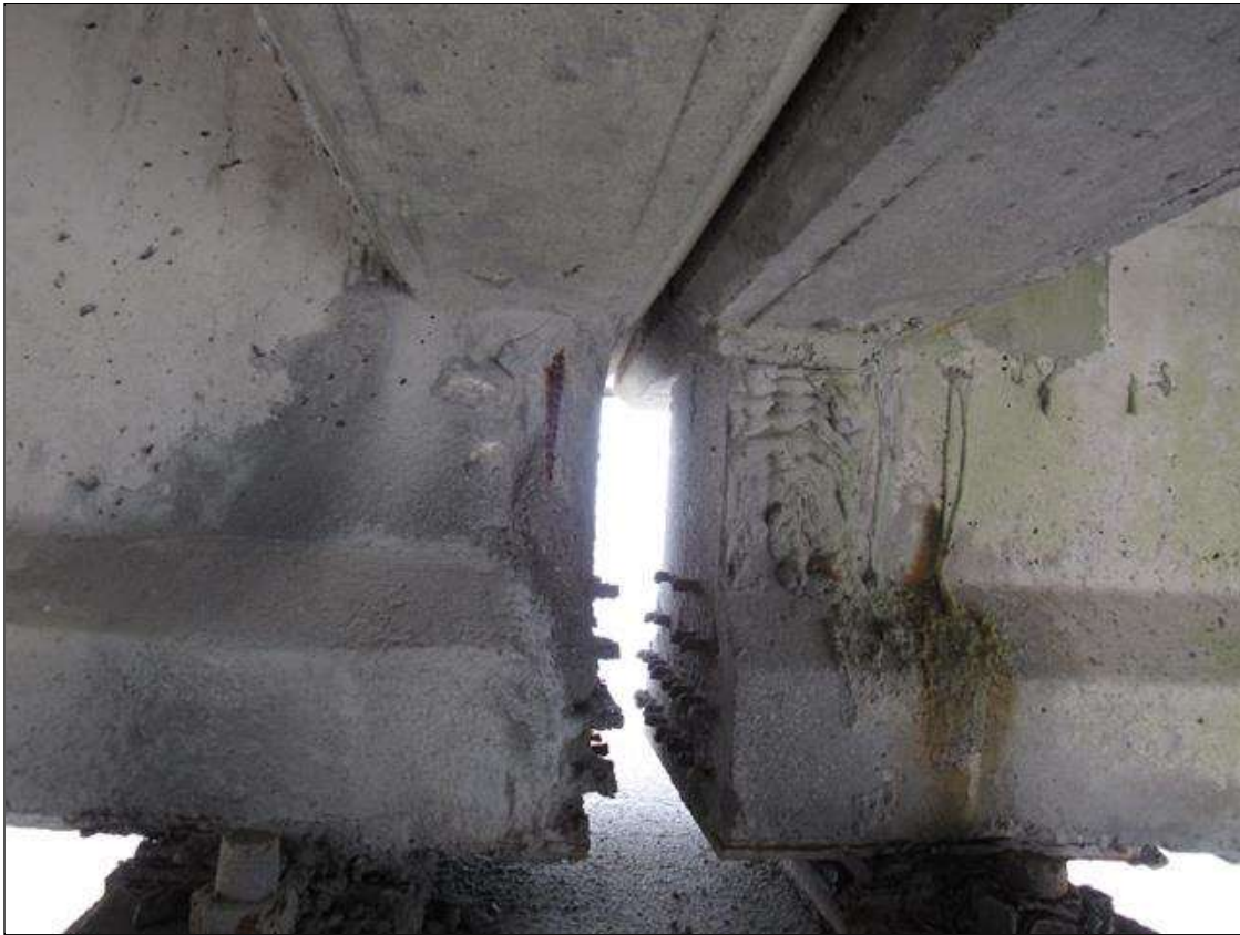
Span 52 Beam 1: 12" X 24" FAILED PATCHED AREA, WITH 6" OF EXPOSED REINFORCING, SOUTH FACE, AT BENT 52.
