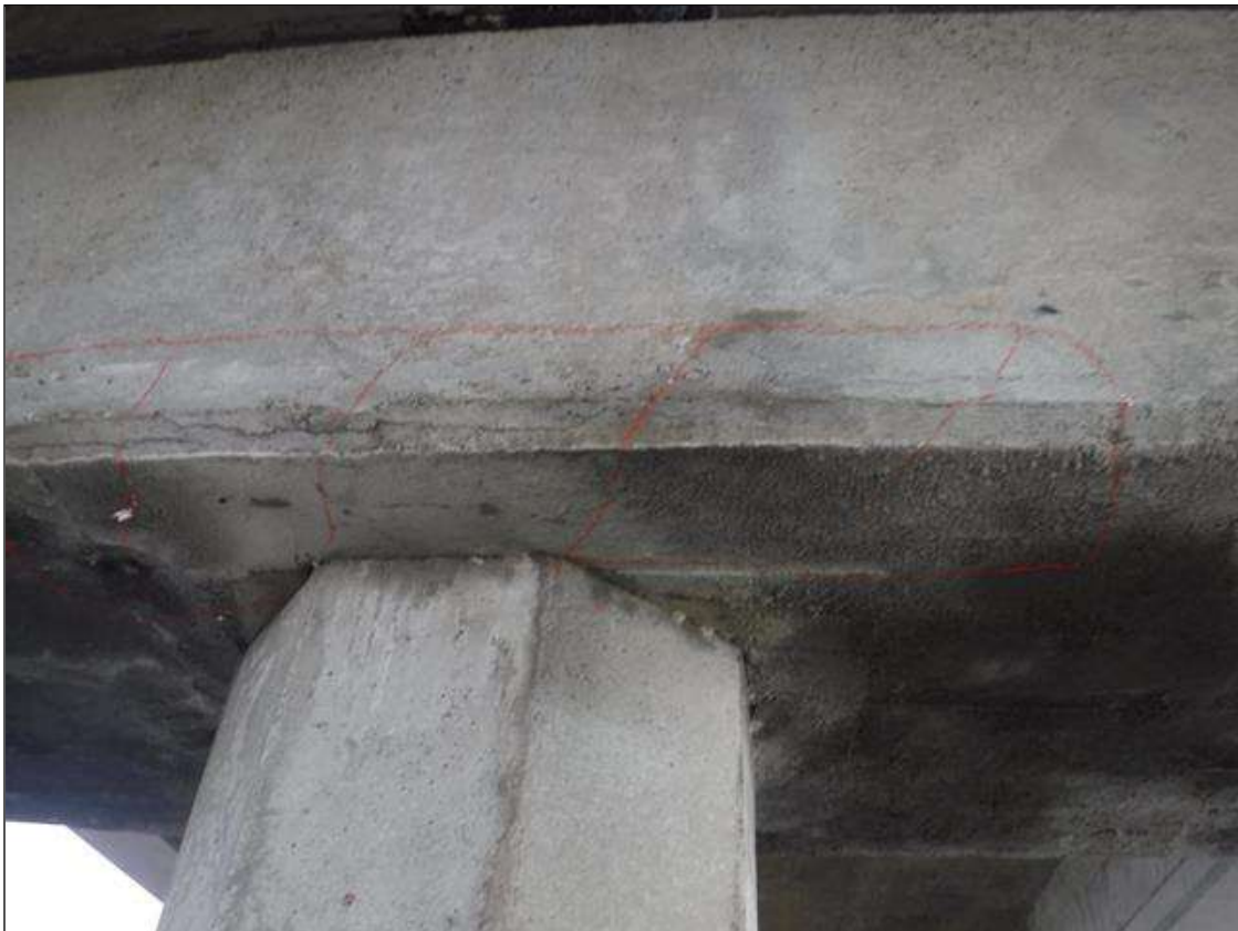
Bent 185 Cap 1: 3' X 6" HIGH X 8" DEEP DELAMINATION ON BOTTOM AND WEST FACE AT PILE 2
