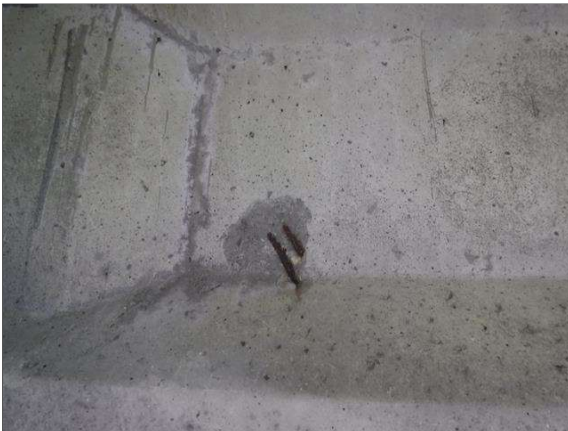
Span 139 Beam 4: (2) 3" DIAMETER X 1/2" SPALL, WITH EXPOSED REBAR, NORTH FACE, 3' FROM BENT 139
