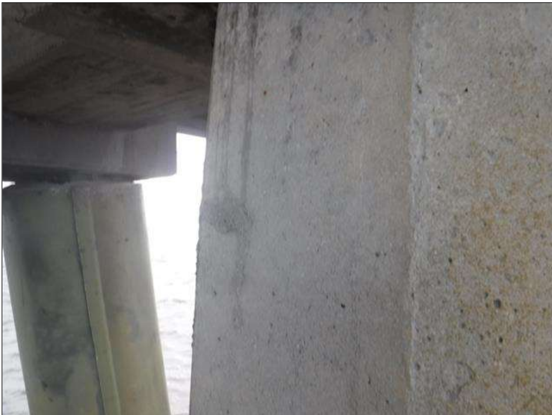
Bent 139 Pile 3: UP TO 2' X 0.009" VERTICAL CRACKS, AT RANDOM THROUGHOUT.
