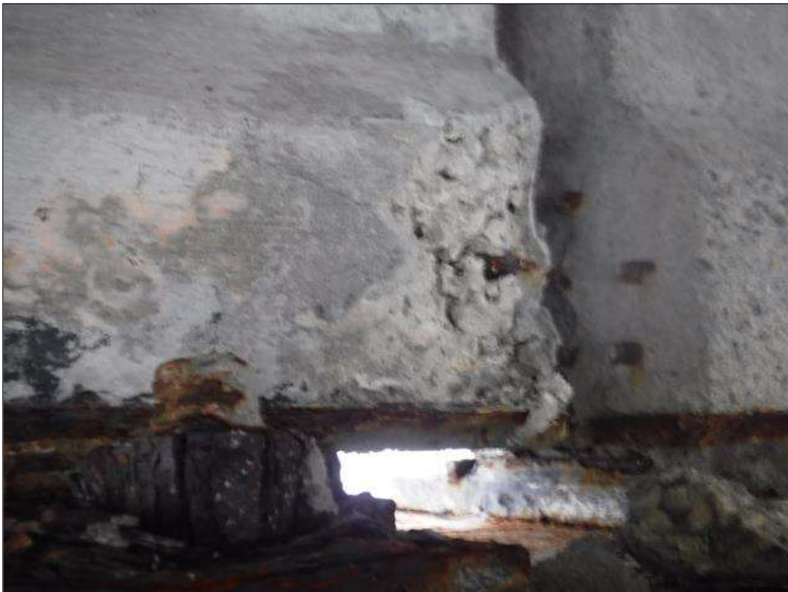
Span 246 Beam 4: (PAR) 6" X 6" X 3" DEEP SPALL WITH EXPOSED STRANDS ON NORTH FACE AT BENT 245
