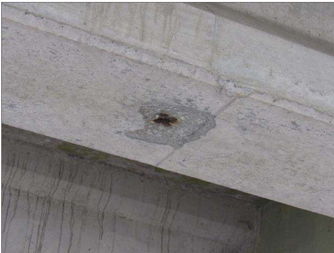
Span 35 Beam 3: 5" DIAMETER X 1/2" DEEP SPALL ON BOTTOM FACE AT MIDSPAN
