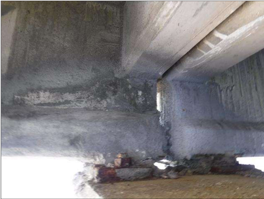
Span 13 Beam 4: 12" X 6" PATCHED AREA ON NORTH FACE AT BENT 12.
