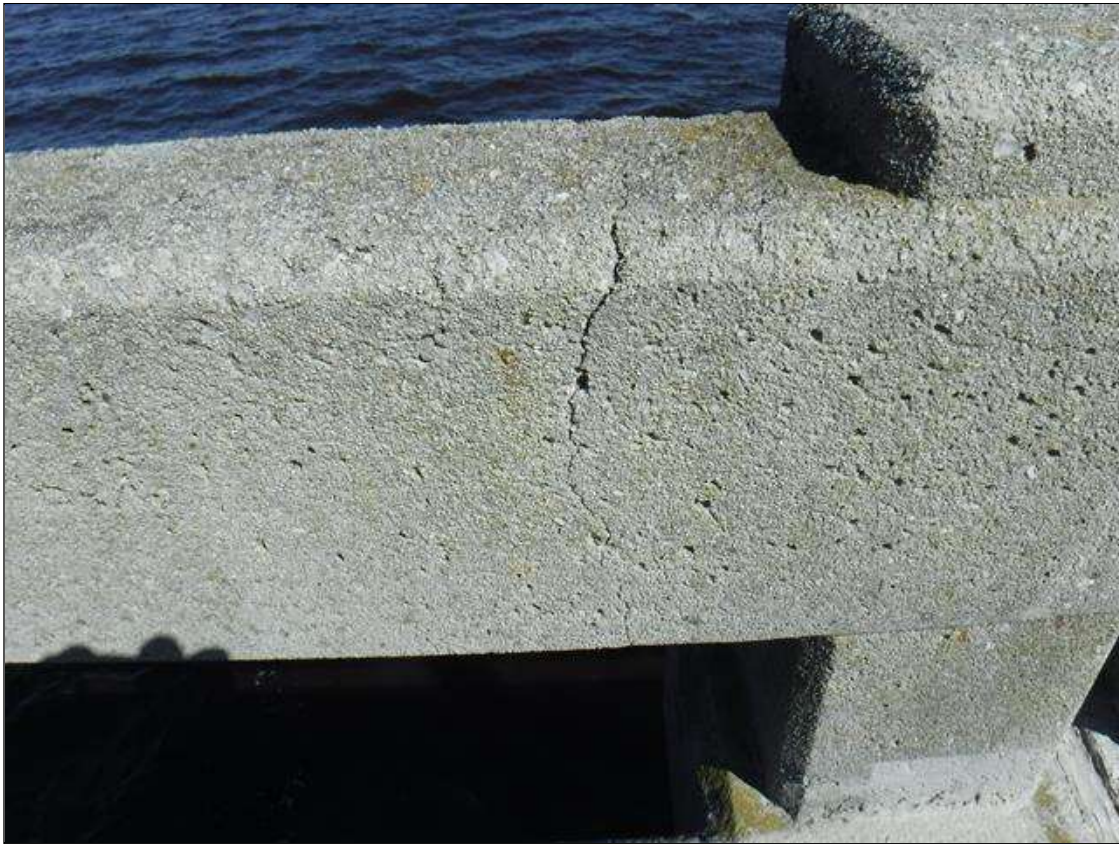
Span 43 Right Bridge Rail: WRAP AROUND CRACK IN RAIL UP TO 1/16" WIDE CRACK LOCATED AT POST 9 AT BENT 43
