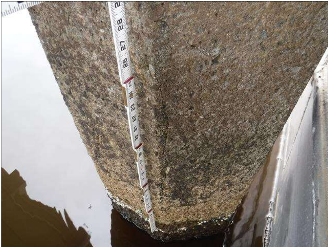
Bent 234 Pile 4: (PAR) (3) UP TO 3' X 0.25" VERTICAL CRACKS, BEGINNING 7' FROM BOTTOM OF CAP, AT RANDOM THROUGHOUT. WITH ADJACENT 3' X 2' DELAMINATION ON NORTH FACE
