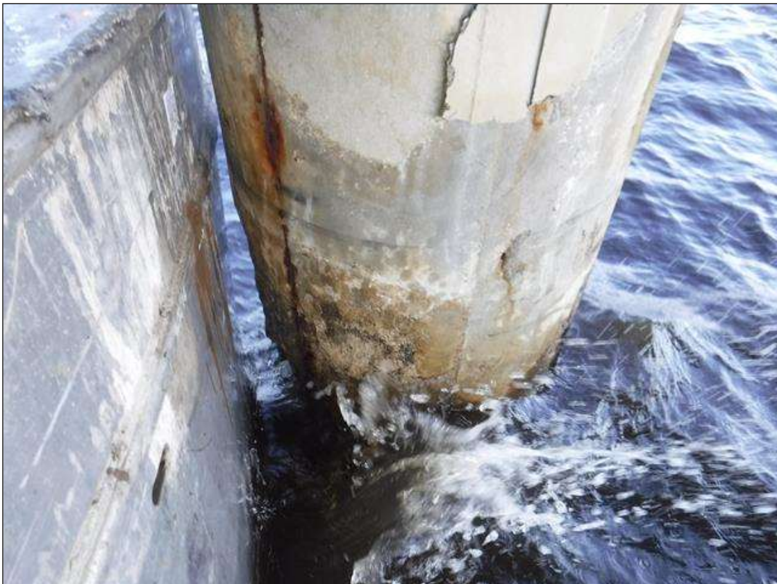
Bent 12 Saved Pile 1: (PAR) 3' X 2' X UP TO 2" SPALL ON PILE JACKET, WITH EXPOSED REINFORCING WITH COMPLETE SECTION LOSS, NORTH FACE, 5' FROM BOTTOM OF CAP AND EXTENDING BELOW WATERLINE.
