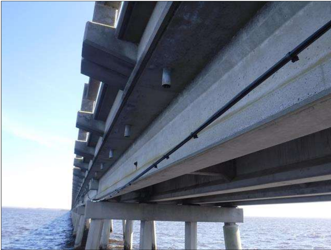
UTILITY HANGING 2' BELOW BEAM 1, SPANS 28 AND 29
