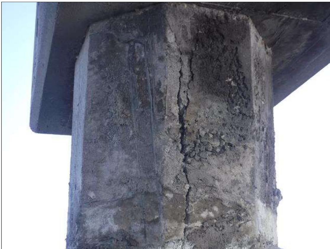
Bent 14 Saved Pile 1: 2' X 1' DELAMINATION ON SOUTH FACE AT BOTTOM OF CAP
