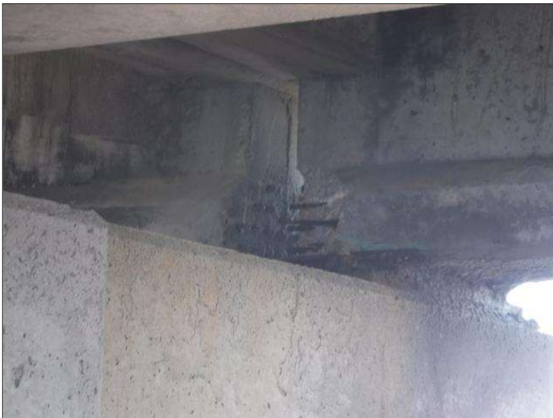
Span 21 Beam 4: (PAR) 12" X 12" X 6" SPALL, WITH EXPOSED PRESTRESSING STRAND, NORTH FACE, AT BENT 21.
