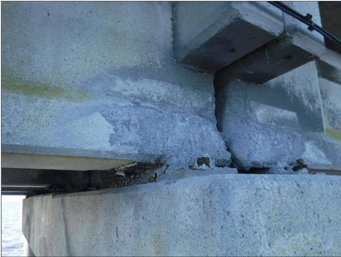
Span 19 Beam 1: 12" X 12" PATCHED AREA, NORTH FACE, AT BENT 18.
