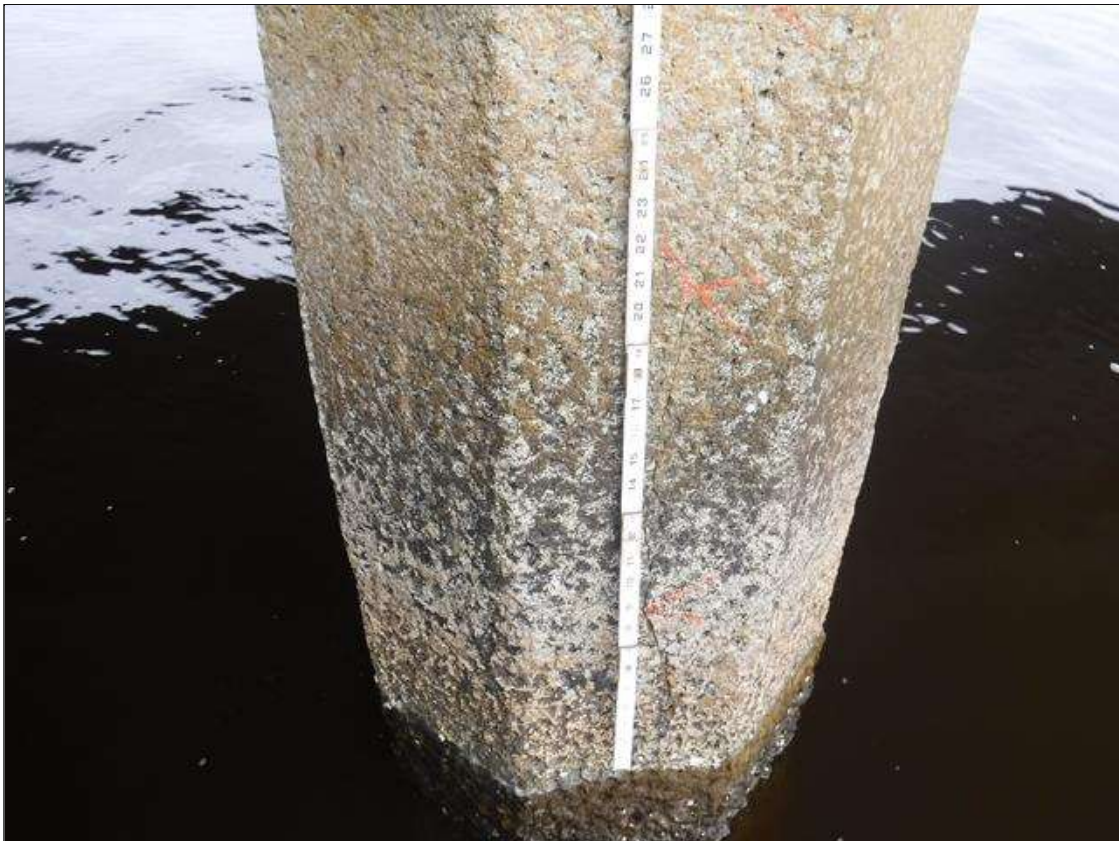
Bent 266 Pile 1: (PAR) HAIRLINE TO 1/16" CRACK, 8' BELOW CAP, DOWN 4', NORTH FACE. SCALING TO 1" DEEP WITH LOOSE AGGREGATE FROM WATERLINE TO MUDLINE.
