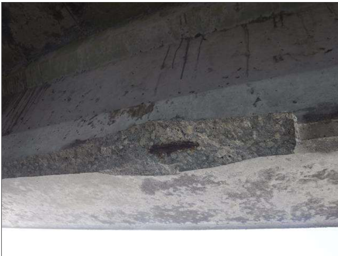
Span 158 Beam 4: (PAR) 3' X 6" X 2" DEEP SPALL WITH EXPOSED STRAND ON BOTTOM LEFT FLANGE 12' FROM BENT 157
