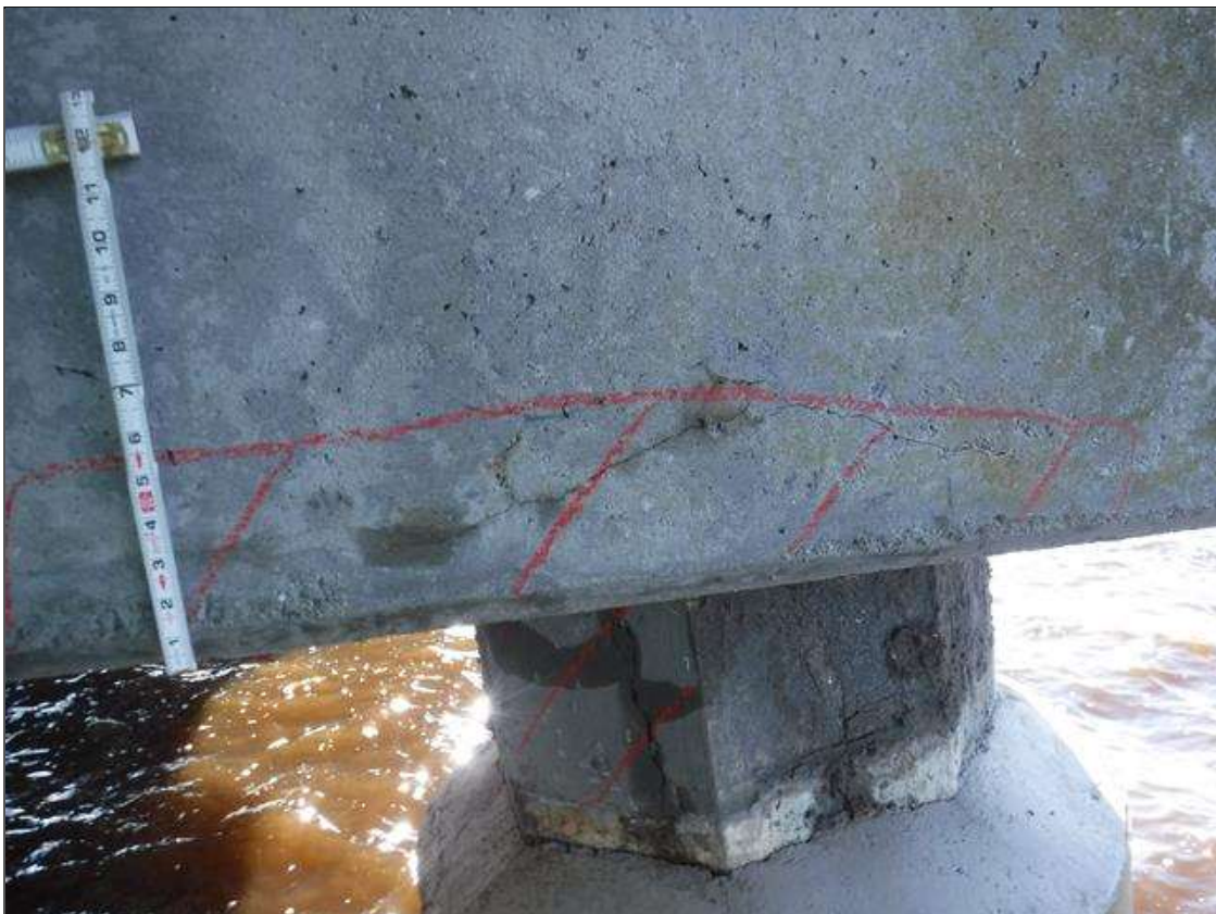
Bent 9 Cap 1: 3' X 8" DELAMINATION, WEST FACE, ABOVE PILE 4.
