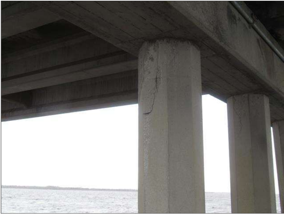
Bent 110 Pile 3: 2' X UP TO 6" X 1 1/2" DEEP SPALL ON SOUTH FACE WITH SURROUNDING DELAMINATION, AT BOTTOM OF CAP, SOUTH FACE.
