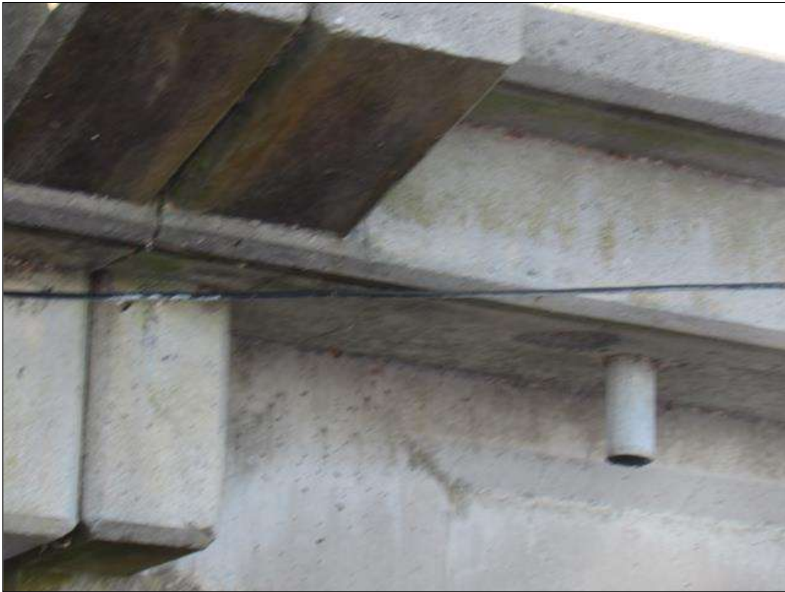
Span 1 Deck: 8" DIAMETER X 1" SPALL, WITH EXPOSED REINFORCING, DECK UNDERSIDE, NORTH OVERHANG, 3' FROM BENT 1.
