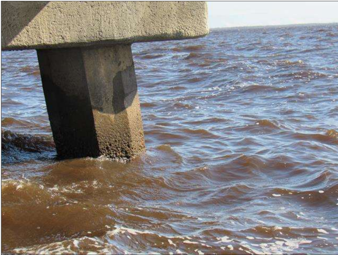
Bent 5 Saved Pile 6: SCALING TO 1" WITH LOOSE AGGREGATE FROM WATERLINE TO MUDLINE
