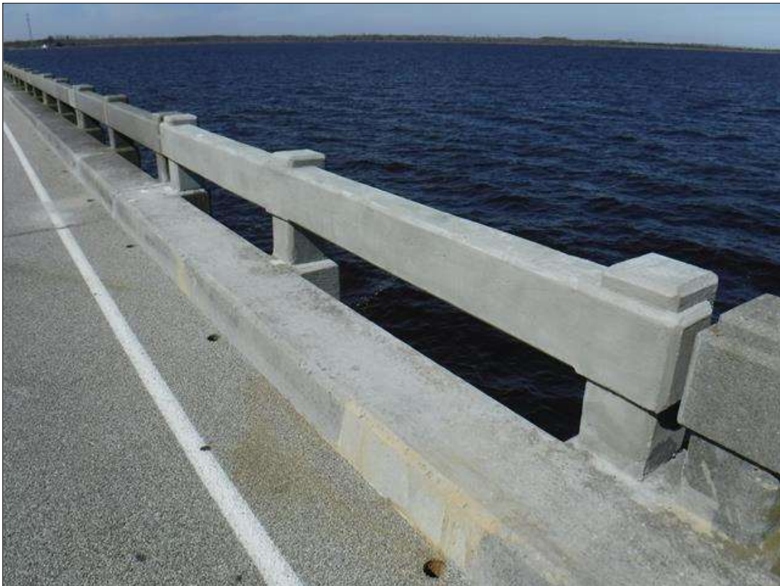
Span 89 Left Bridge Rail: 12' PATCHED LENGTH OF RAIL LOCATED IN FIRST SECTION OF RAIL FROM POST 1 TO POST3
