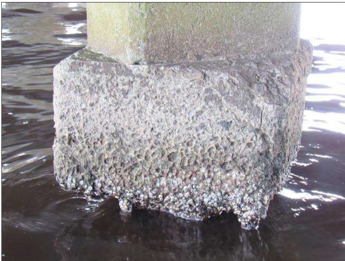
Bent 278 Pile 2: (PAR) 8' X 1' X 8" DEEP SPALL WITH EXPOSED REINFORCING LOCATED ON ALL FACES
