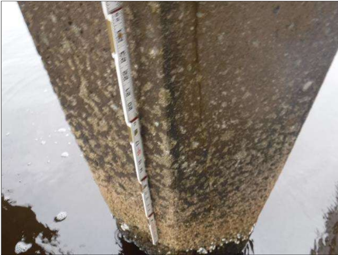
Bent 248 Pile 4: (PAR) 3' X 1/16" VERTICAL CRACK WITH SURROUNDING 36" X 8" DELAMINATION ON NORTH FACE, 7' FROM BOTTOM OF CAP.
