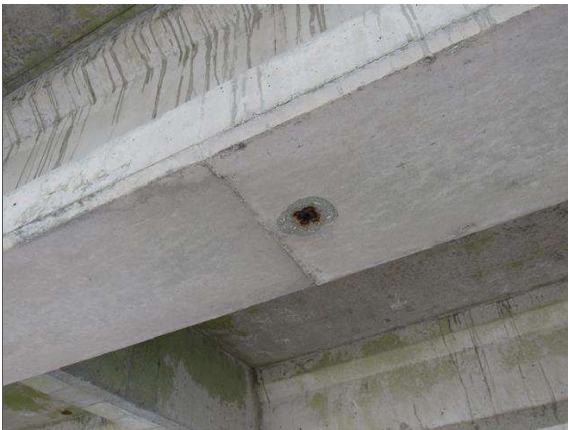
Span 49 Beam 3: 3" DIAMETER SPALL, 5' EAST OF MID SPAN
