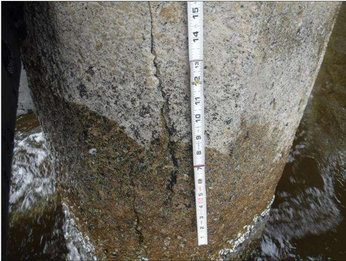
Bent 183 Pile 6: (PAR) HAIRLINE TO 1/8" CRACKS, 8' BELOW CAP, DOWN 4', MULTIPLE FACES. SCALING TO 1" DEEP WITH LOOSE AGGREGATE FROM WATERLINE TO MUDLINE.
