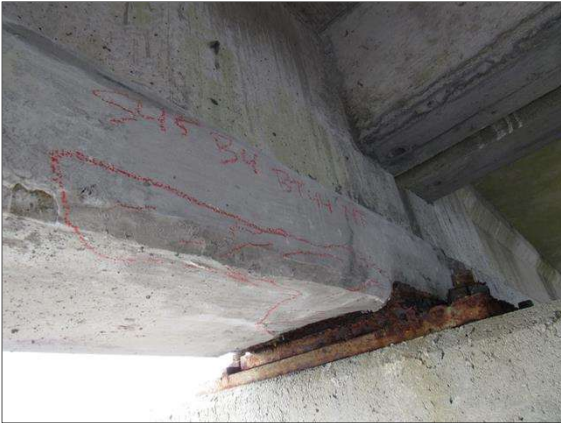
Span 45 Beam 4: 3' X UP TO 9" PATCHED AREA WITH 22" X 11" OF DELAMINATION, BOTTOM FACE, EXTENDING 10" ONTO NORTH FACE, AT BENT 44.
