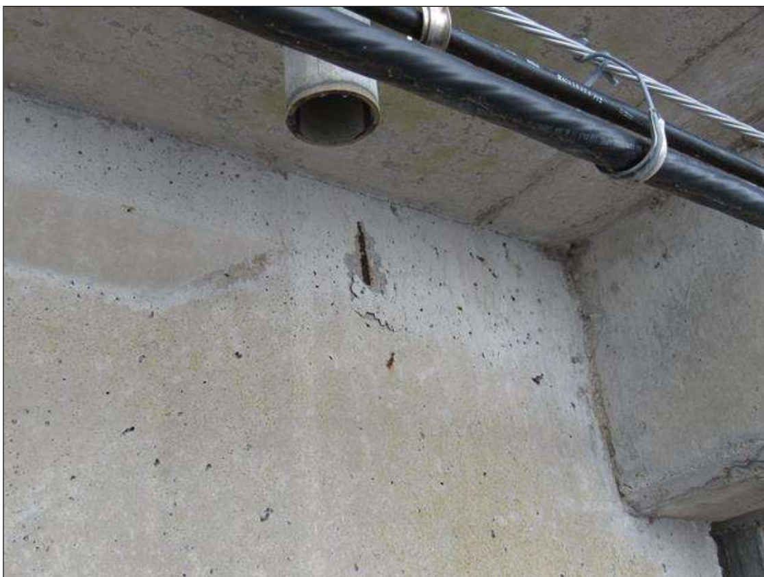
Span 61 Beam 4: 2" X 4" X 1/8" SPALL, WITH EXPOSED REINFORCING, TOP OF SOUTH FACE, 2' FROM BENT 61.
