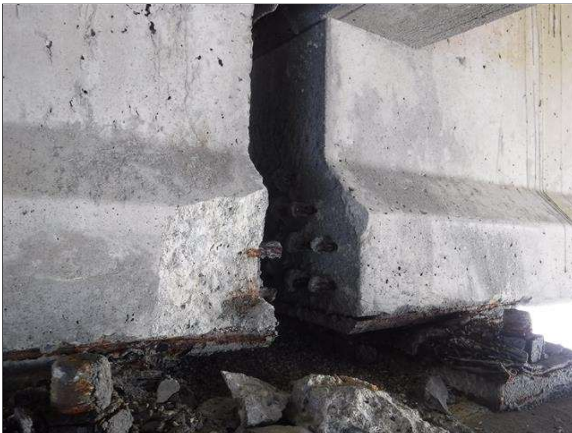
Span 74 Beam 3: (PAR) 6" X 6" X 3" DEEP SPALL WITH EXPOSED STRAND ON SOUTH FACE AT BENT 74
