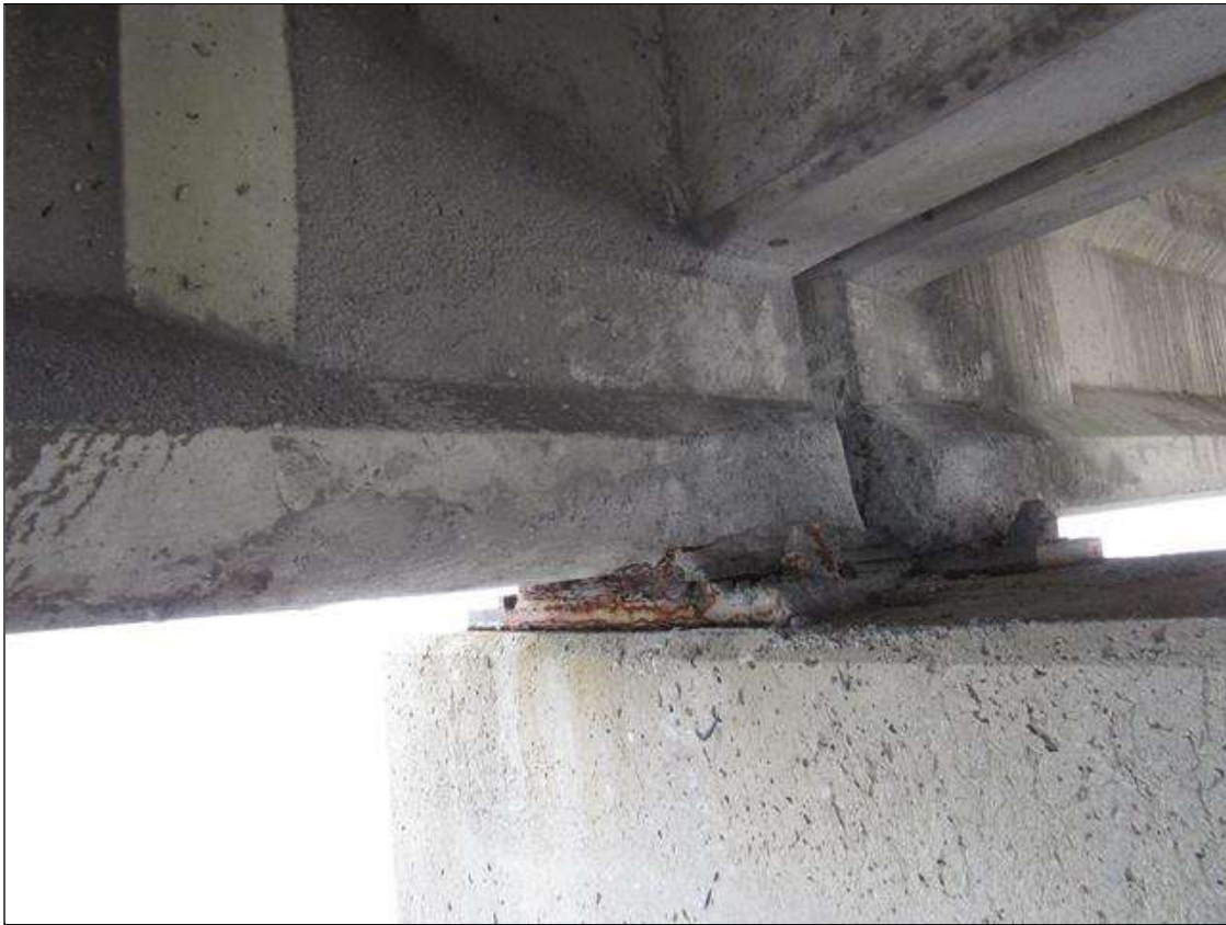
Span 37 Beam 1: 2' X UP TO 6" FAILED PATCHED AREA, BOTTOM FACE, EXTENDING 10" ONTO SOUTH FACE, AT BENT 37.
