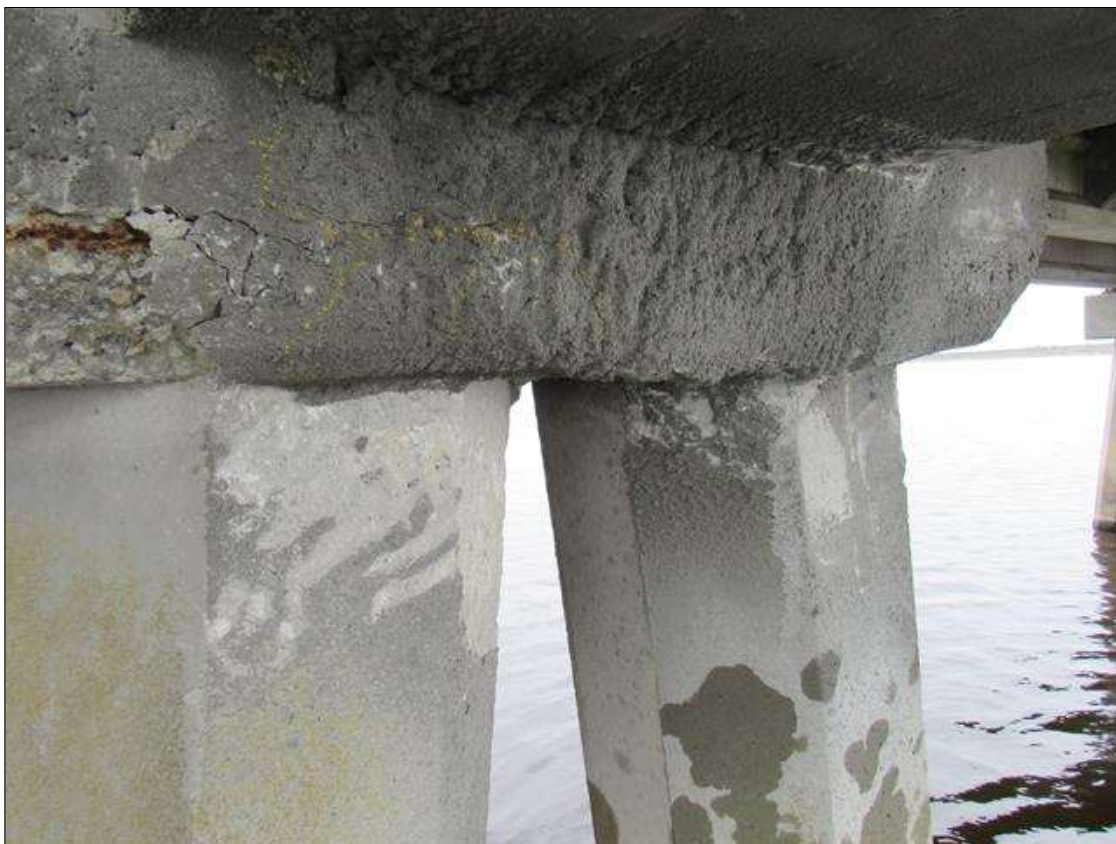
Bent 45 Cap 1: 14" X 8" WIDE DELAMINATION ON EAST FACE LOCATED LEFT OF PILE 3
