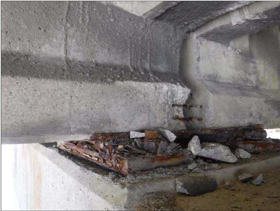
Span 114 Beam 3: (PAR) 8" X 6" X 2" DEEP SPALL WITH EXPOSED STRANDS ON SOUTH FACE AT BENT 114
