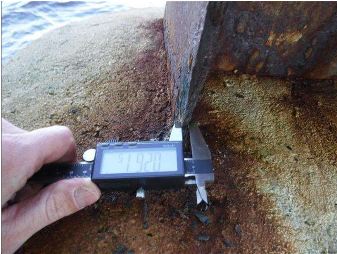
Bent 120 Saved Pile 1: (PAR) 2" X 1" AREA OF CORROSION WITH SECTION LOSS ON NEAR RIGHT FLANGE, 0.26" REMAINING FLANGE THICKNESS MEASURED ABOVE CONCRETE JACKET
