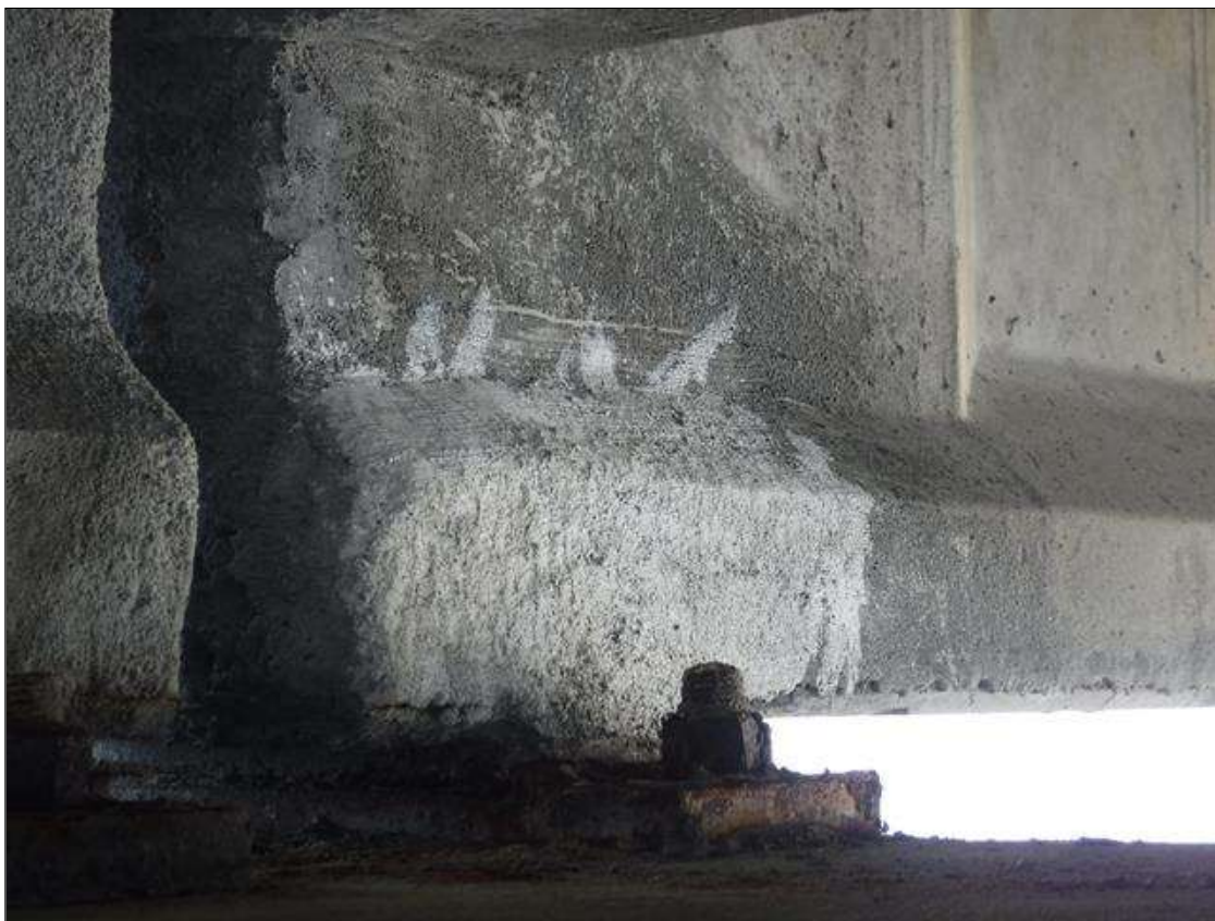
Span 155 Beam 1: 1' X 1' PATCHED AREA, SOUTH FACE, AT BENT 154.
