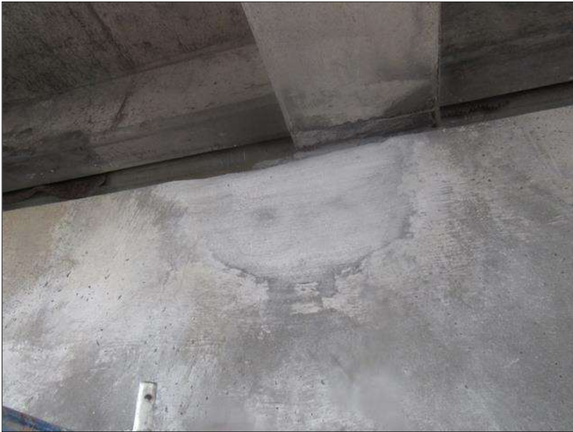
Bent 74 Cap 1: 36" X 18" PATCHED AREA, EAST FACE, BELOW BEAM 3.
