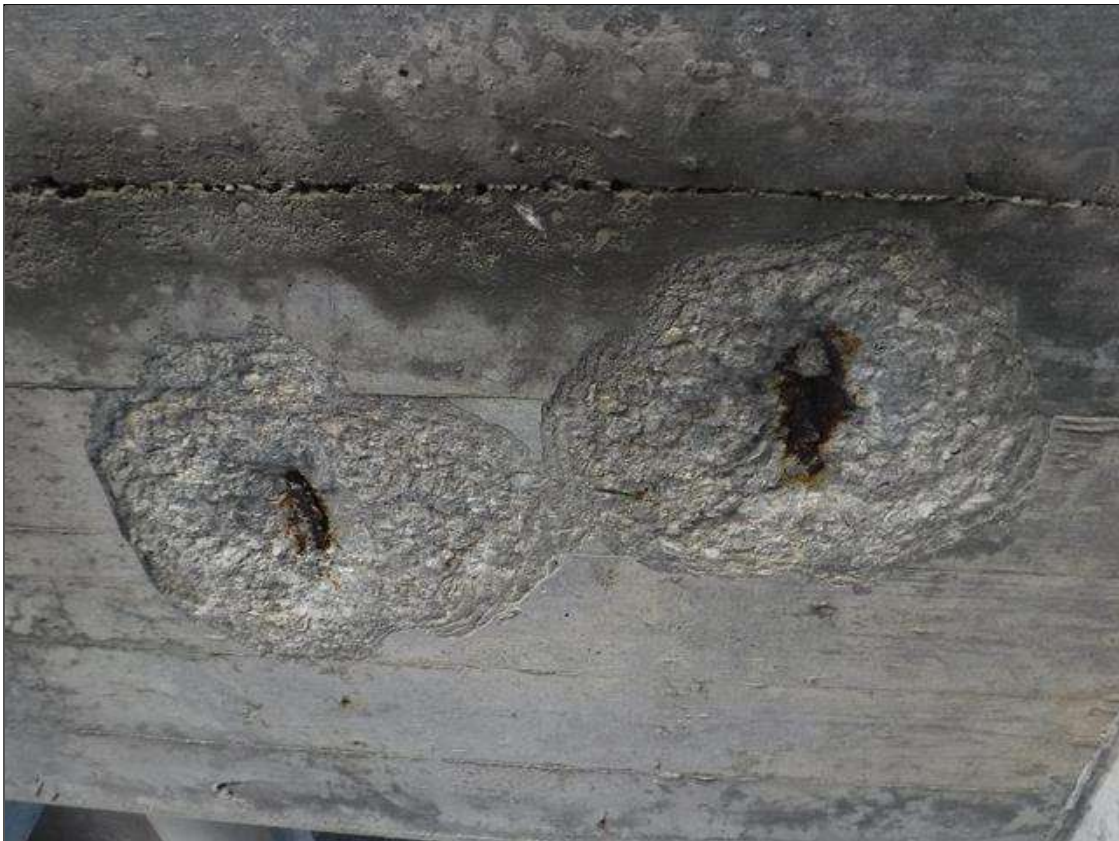
Bent 207 Cap 1: (PAR) (2) 12" DIAMETER SPALLS WITH EXPOSED REBAR ON BOTTOM OF CAP AT MIDSPAN. REBAR HAS 10% SECTION LOSS
