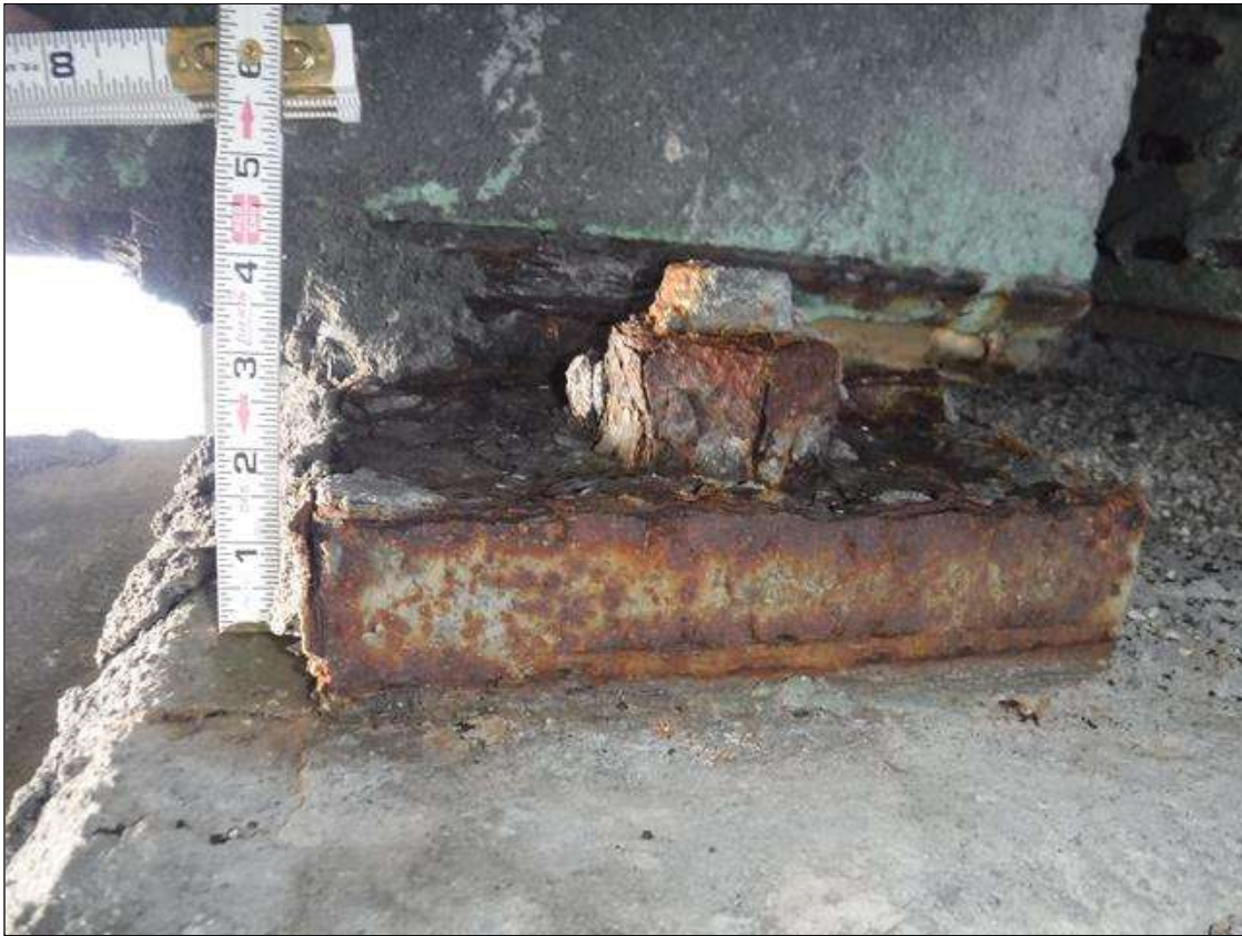
Span 10 Beam 2 Near Bearing: CORROSION WITH LESS THAN 1/16" LOSS. (2" REMAINING).
