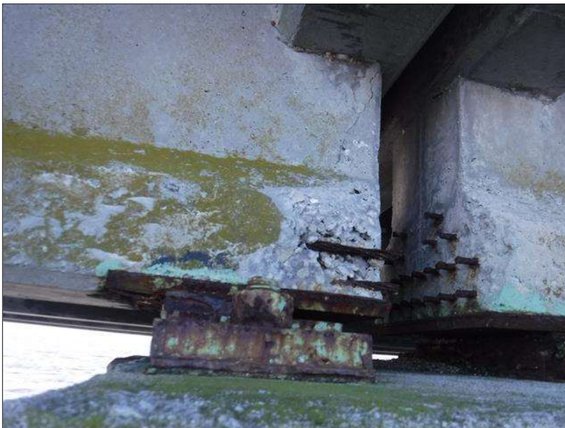
Span 14 Beam 1: (PAR) 8" X 8" X 2" SPALL, WITH EXPOSED PRESTRESSING STRAND, NORTH FACE, AT BENT 13.
