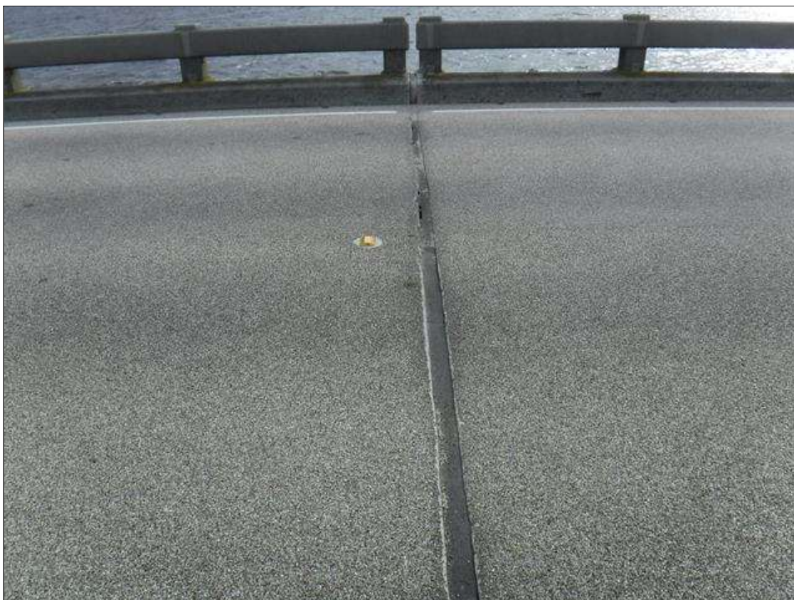
Expansion Joint 246 : FULL LENGTH SEAL DAMAGE WITH LOSS OF ADHESION LOCATED AT BENT 246
