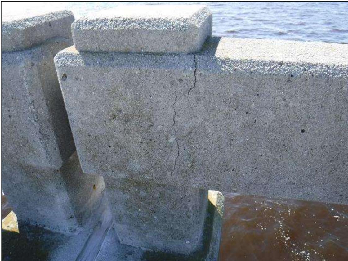
Span 42 Right Bridge Rail: 12" VERTICAL CRACK UP 1/16" WIDE ON LEFT FACE LOCATED AT POST 9 AT BENT
