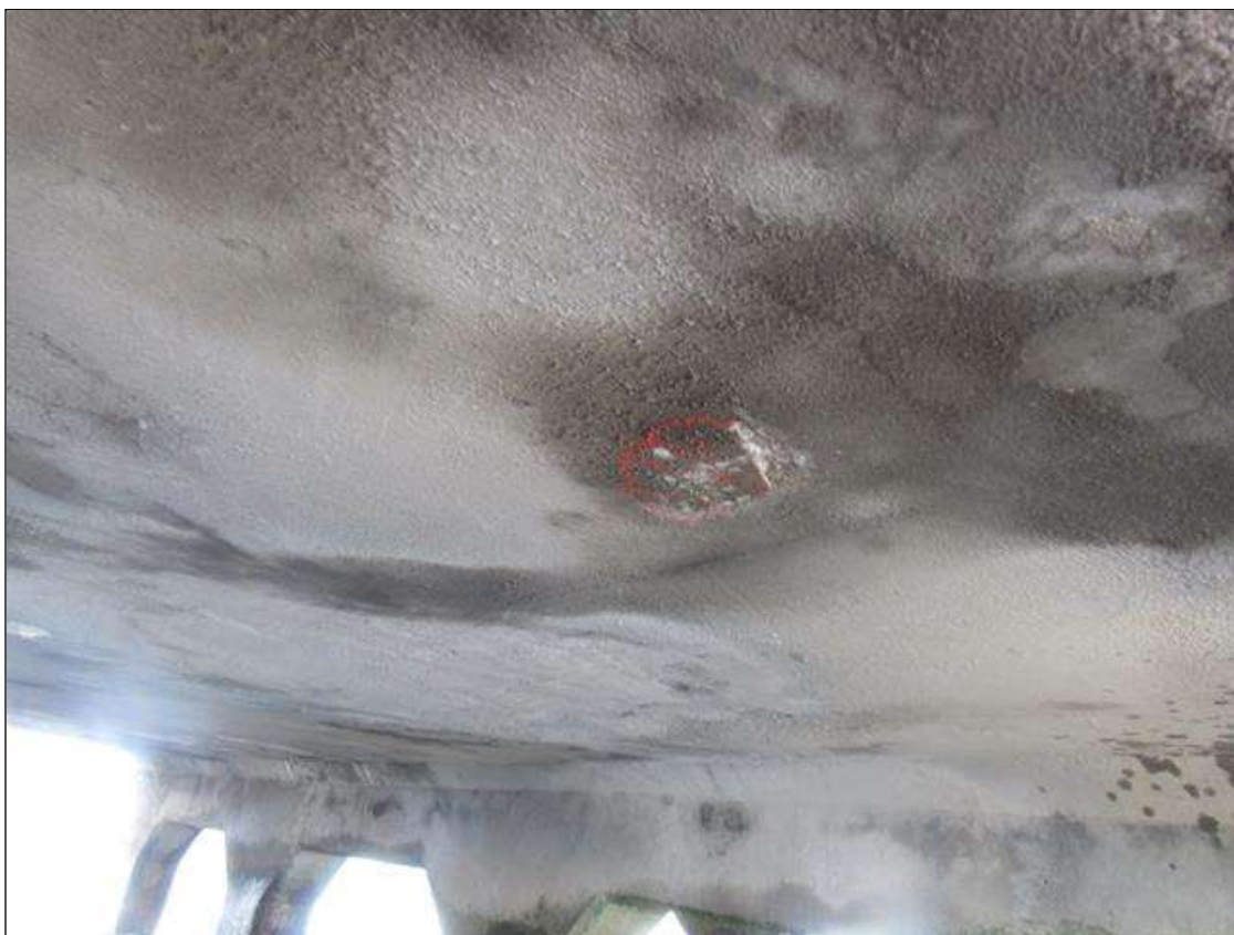
Span 295 Deck: 8" DIAMETER DELAMINATION ON BOTTOM FACE LOCATED 3' FROM LEFT EDGE AT MIDSPAN
