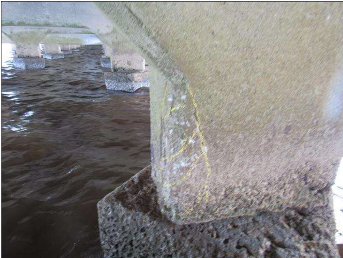
Bent 280 Pile 3: 14" X 3" X 3" DELAMINATION, NORTHWEST CORNER, 1' FROM BOTTOM OF CAP.
