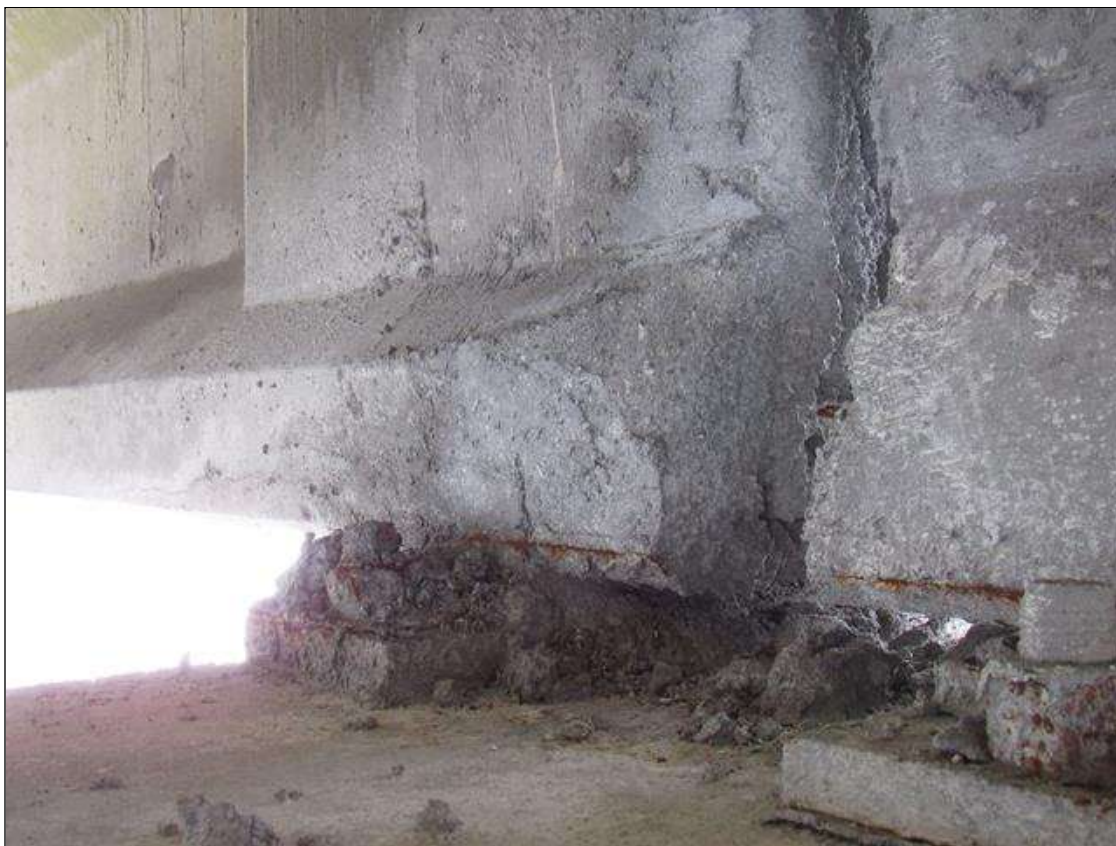
Span 40 Beam 4: 9" X 18" PATCHED AREA, NORTH FACE, AT BENT 39.
