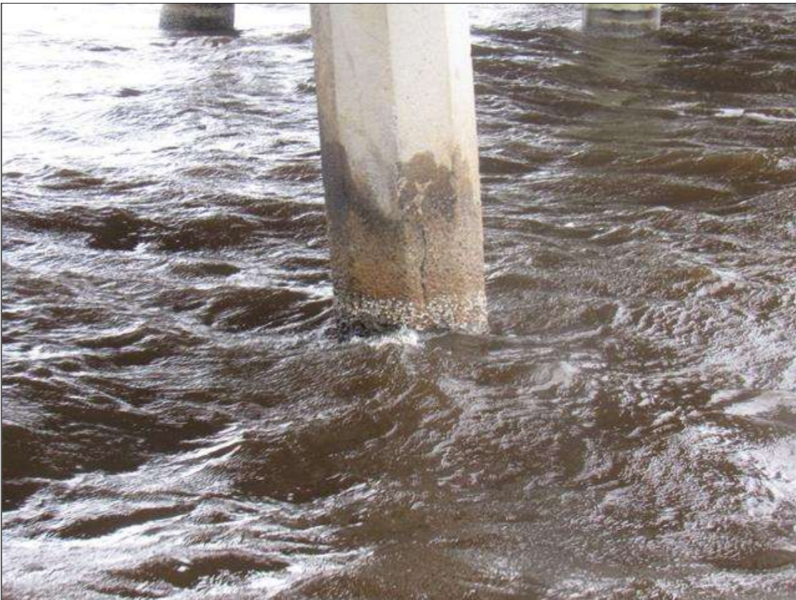
Bent 98 Pile 4: (PAR) 2' X 0.012" VERTICAL CRACK, SOUTH FACE, 9' FROM BOTTOM OF CAP, WITH ADJACENT 2' X 1' DELAMINATION.
