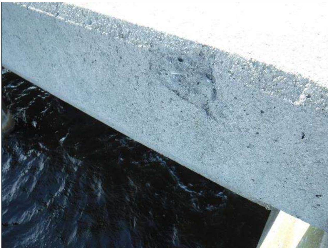
Span 191 Left Bridge Rail: 4" DIAMETER X 1" DEEP SPALL ON LEFT FACE LOCATED ON RAILING 1' PAST POST 5
