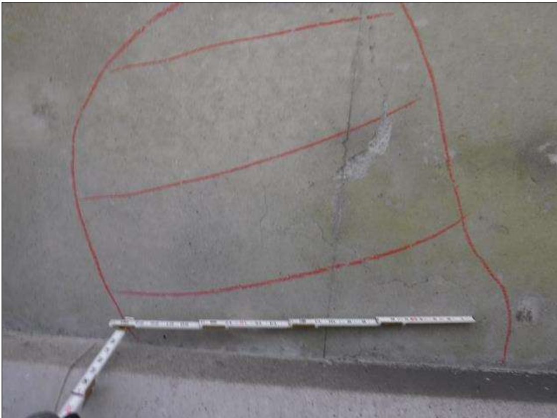
Span 228 Deck: 2' DIAMETER DELAMINATION ON UNDERSIDE OF DECK BETWEEN BEAM 2 AND 3, 10' FROM BENT 227
