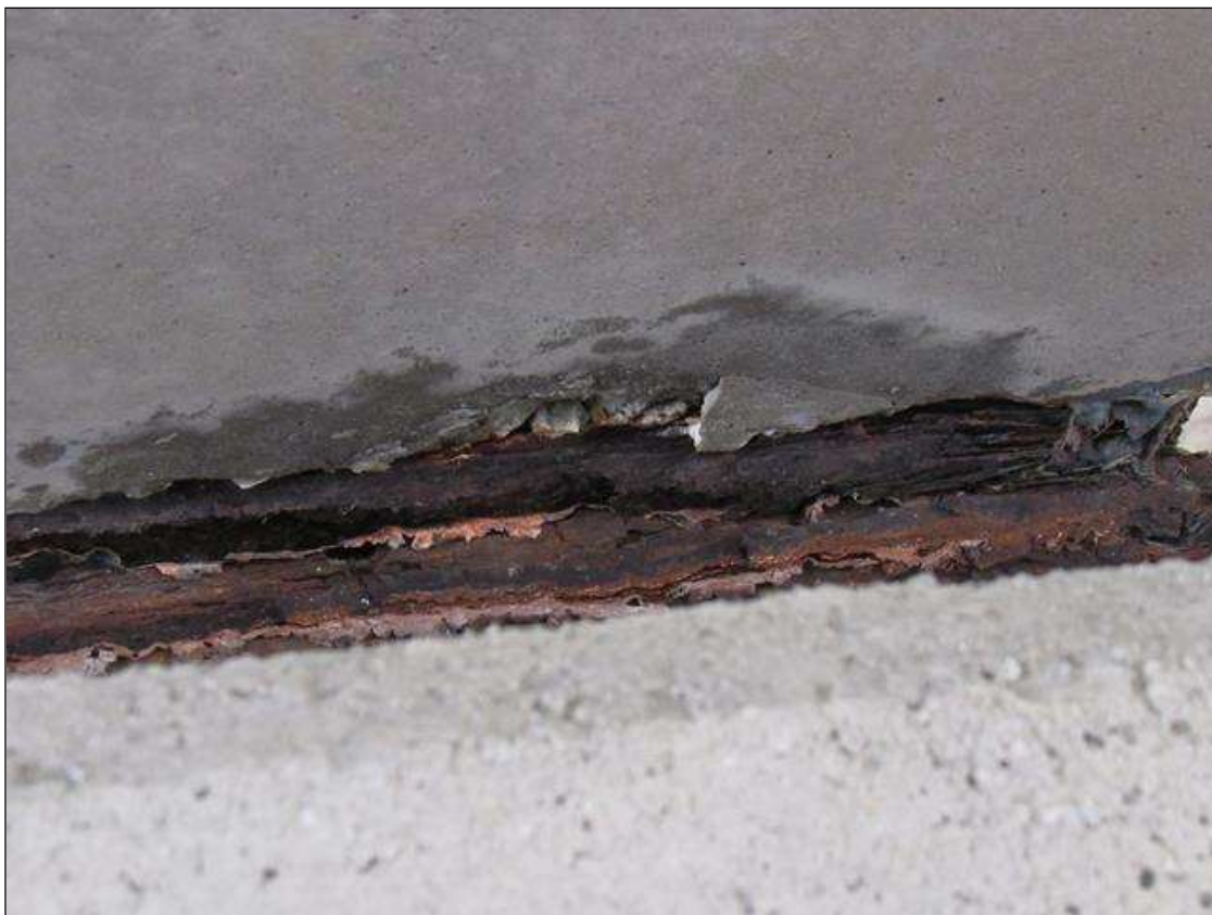
Span 49 Beam 2: 6" LONG X 1" HIGH SHALLOW SPALL WITH DELAMINATION ON BOTTOM EDGE AT BENT 49 BEARING
