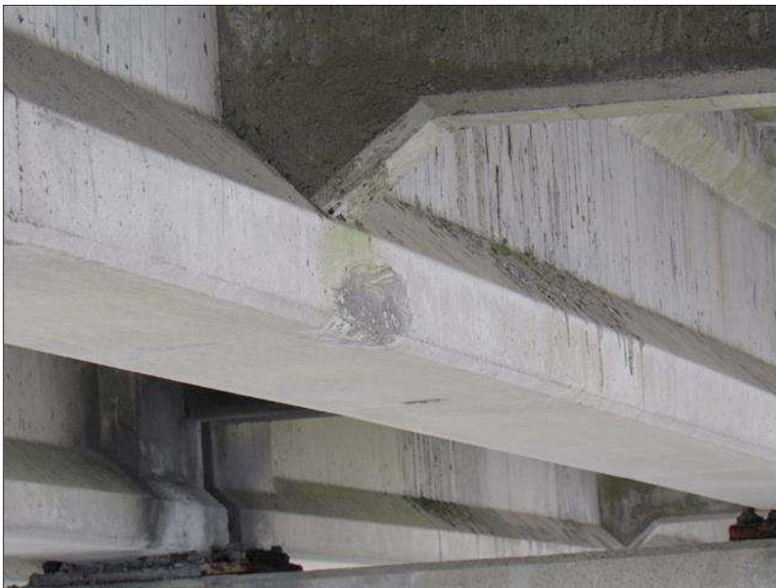
Span 55 Beam 2: 18" X 12" PATCHED AREA, NORTH FACE, AT BENT 55.
