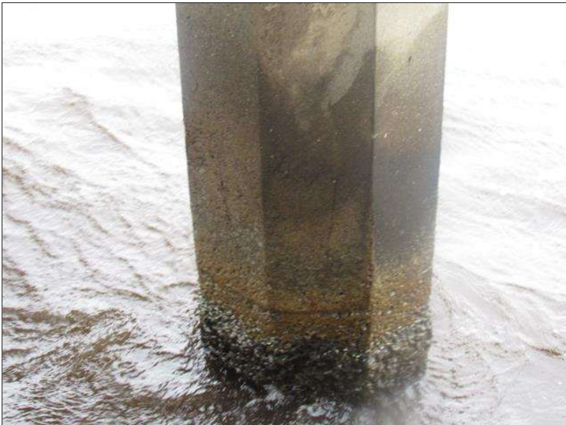
Bent 74 Pile 1: (PAR) (4) UP TO 3' X 0.06" VERTICAL CRACKS WITH SURROUNDING 3' X 1' DELAMINATION, BEGINNING 8' FROM BOTTOM OF CAP, AT RANDOM THROUGHOUT.
