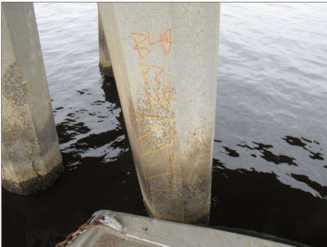
Bent 49 Saved Pile 2: 4' X 11" DELAMINATION WITH SURROUNDING HAIRLINE VERTICAL CRACK, NORTH FACE, BEGINNING 6' FROM BOTTOM OF CAP.
