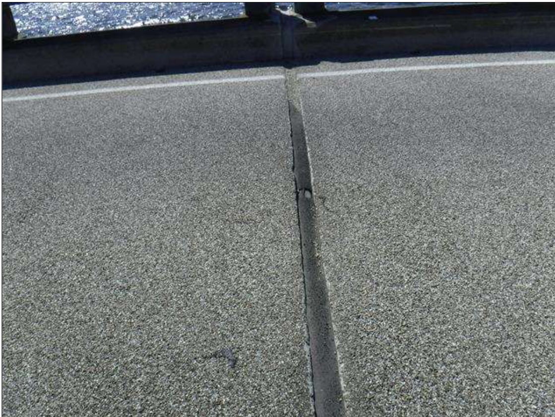
Expansion Joint 82 : 2' SEAL DAMAGE WITH LOSS OF ADHESION LOCATED IN RIGHT LANE 4' FROM RIGHT SHOULDER
