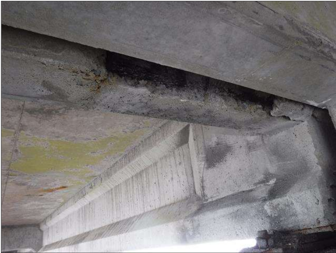
Span 89 Beam 1: (PAR) 3' X 3" X 6" SPALL WITH EXPOSED REBAR IN BAY 1 DIAPHRAGM AT BENT 88
