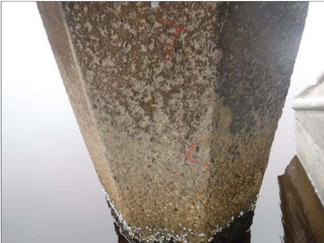
Bent 238 Pile 1: (PAR) UP TO 5' X 0.03" VERTICAL CRACKS, EAST FACE, BEGINNING 5' FROM BOTTOM OF CAP.
