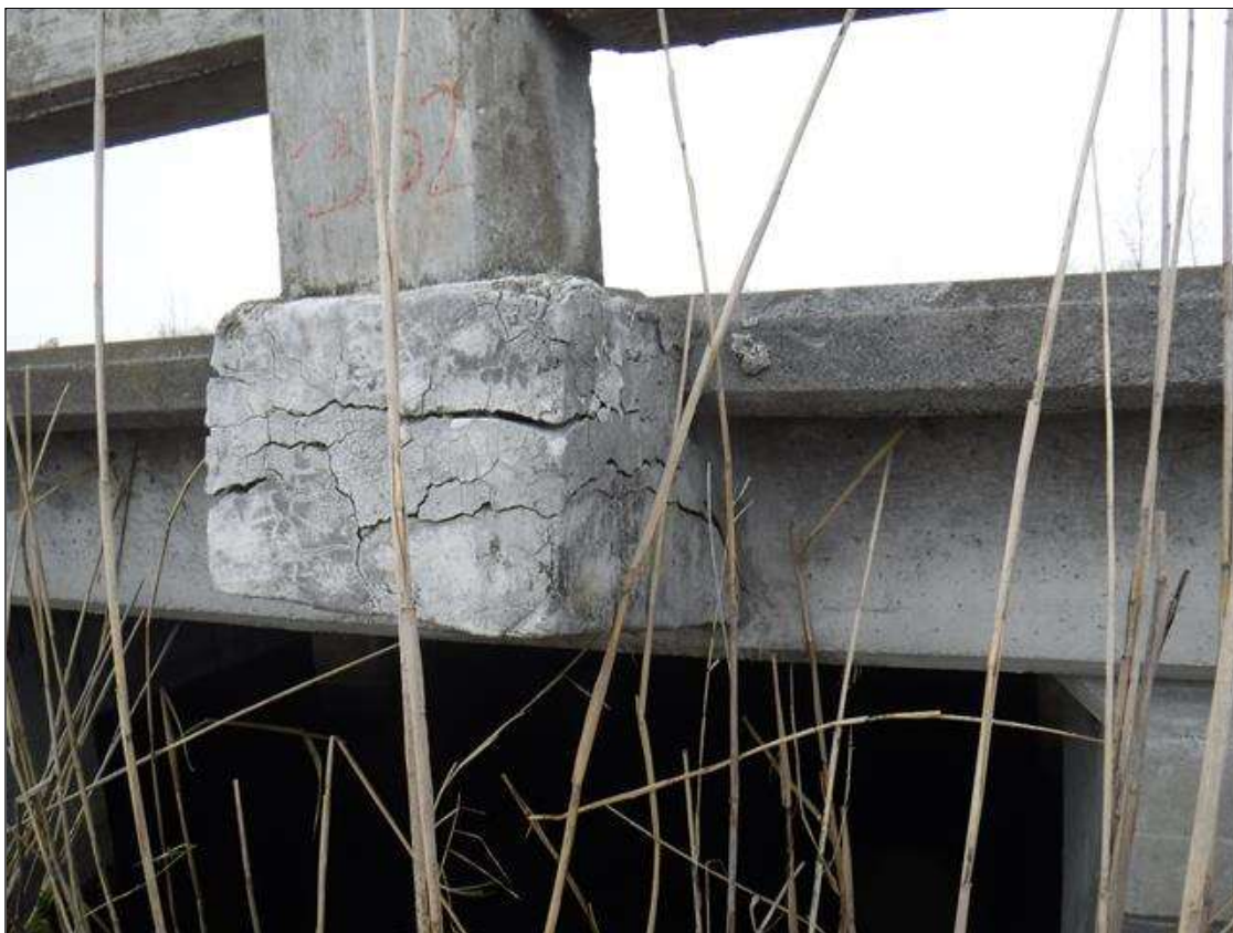
Span 332 Right Bridge Rail: (PAR) 14" X 11" X 23" DELAMINATION AT BOTTOM RIGHT CORNER ON OUTSIDE EDGE OF POST AT MID SPAN
