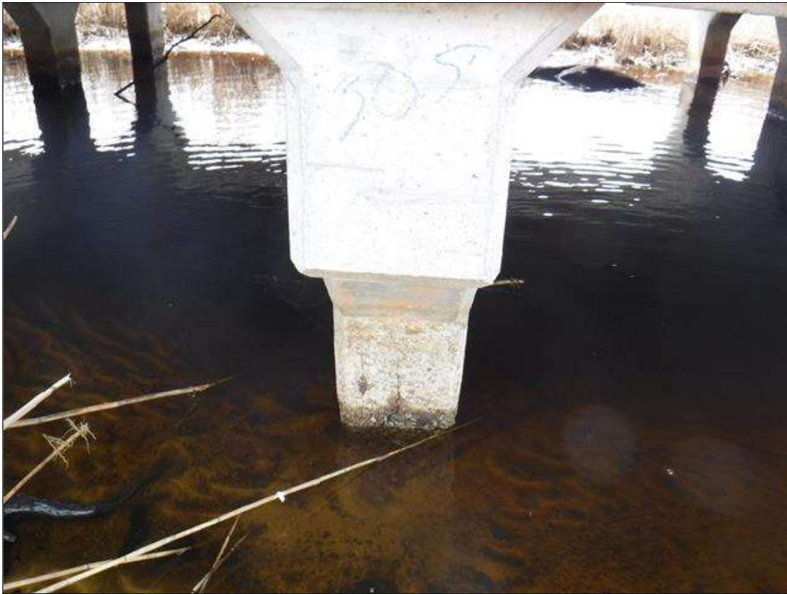
Bent 305 Pile 1: (2) 2' X UP TO 1/16" WIDE VERTICAL CRACKS ON SOUTH FACE LOCATED ON PILE 1
