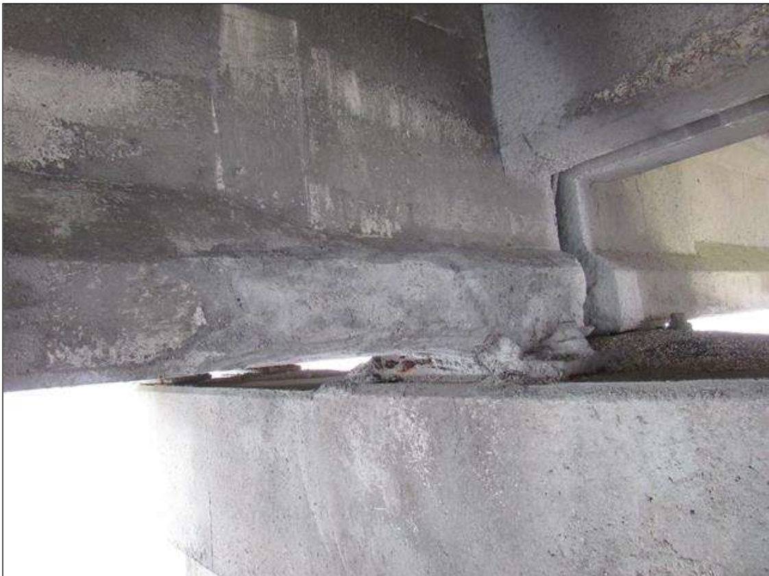
Span 38 Beam 2: 4' X UP TO 8" PATCHED AREA, BOTTOM FACE, EXTENDING 10" ONTO NORTH AND SOUTH FACES, AT BENT 38.
