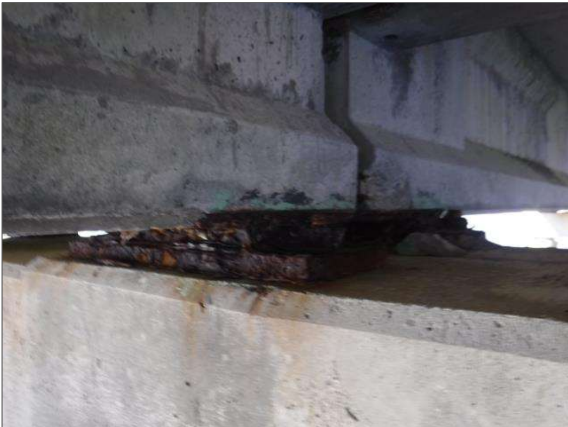
Span 19 Beam 3 Near Bearing: CORROSION WITH LESS THAN 1/16" LOSS. (2" REMAINING).
