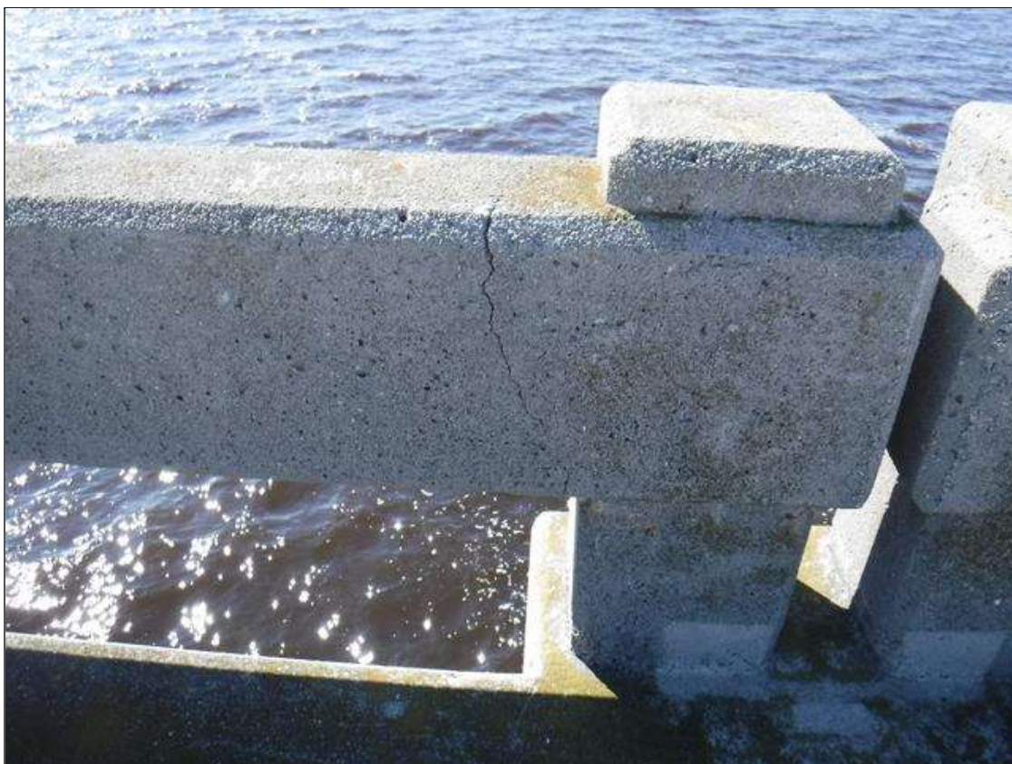
Span 43 Right Bridge Rail: (4) UP TO 1/16" WRAPAROUND CRACKS, AT RANDOM THROUGHOUT
