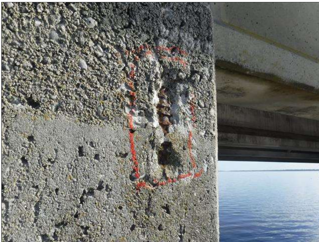
Bent 211 Cap 1: 6" X 3" X 3/4" SPALL, WITH EXPOSED PRIMARY REINFORCING, SOUTH FACE.
