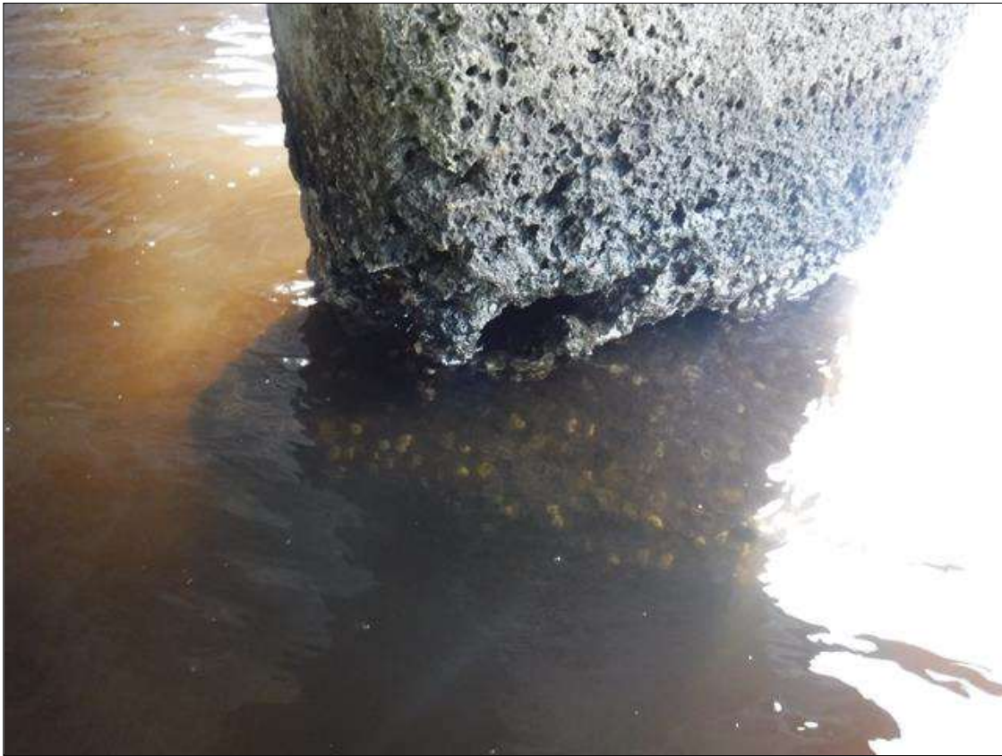
Bent 298 Pile 4: (PAR) 6" DEEP X 8" HIGH X FULL WIDTH SPALL WITH EXPOSED REBAR WITH 25% SECTION LOSS AROUND BASE OF COLUMN AND TOP OF FOOTING
