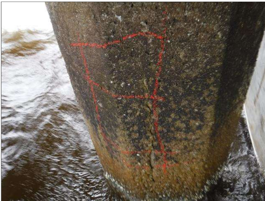
Bent 194 Pile 3: 3' X 1' DELAMINATION, EAST FACE, 7' BELOW BOTTOM OF CAP, EXTENDING BELOW WATERLINE.
