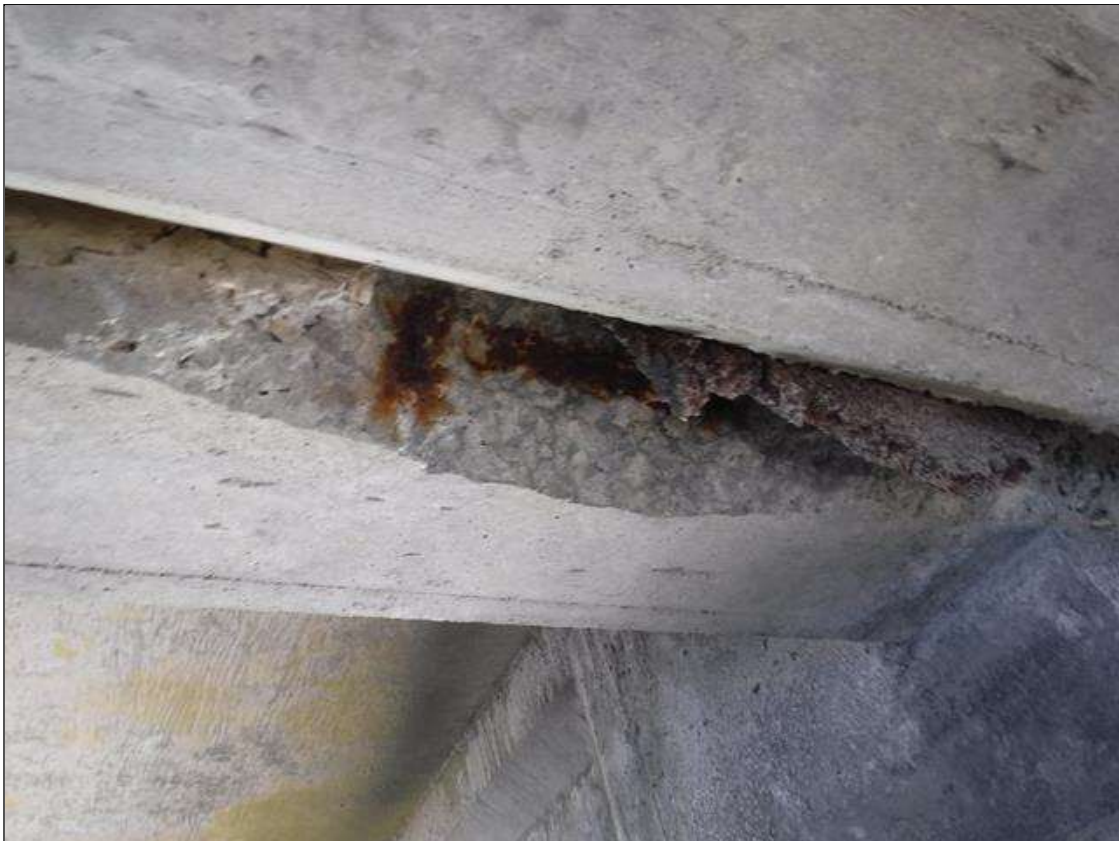
Span 223 Beam 3: (PAR) 3' X 10" X 4" DEEP SPALL WITH EXPOSED REINFORCEMENT IN END DIAPHRAGM BETWEEN BEAM 3 AND 4 AT BENT 222
