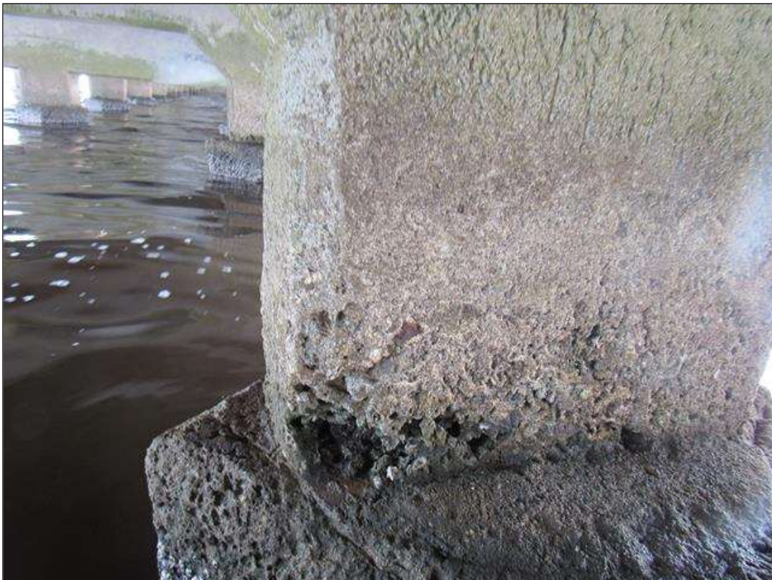
Bent 281 Pile 3: 4" X 4" X 4" DEEP SPALL ON WEST FACE AT COLUMN FOOTING INTERFACE
