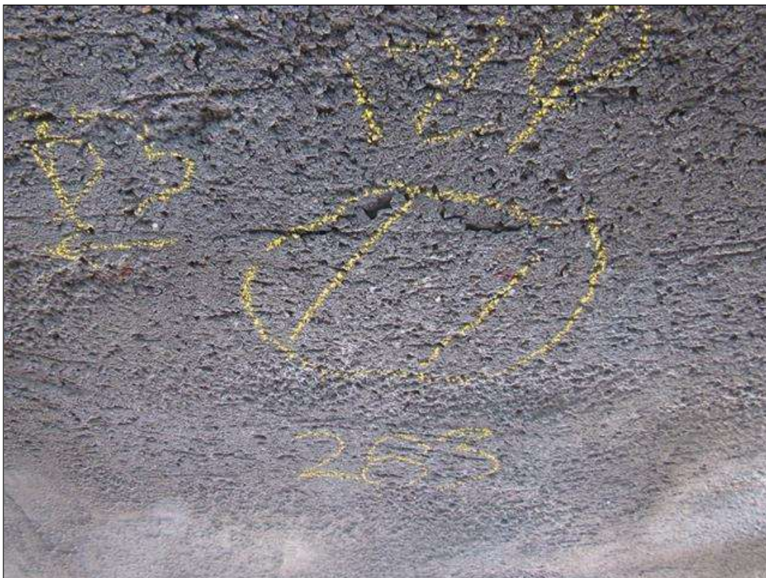
Span 283 Deck: 12" DIAMETER DELAMINATION ON BOTTOM FACE AT MID-SPAN NEAR PILE 3
