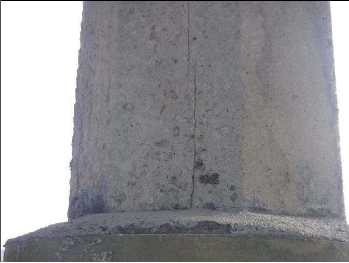
Bent 131 Pile 4: (PAR) UP TO 3' X 0.0625" VERTICAL CRACKS, AT RANDOM THROUGHOUT WEST FACE.
