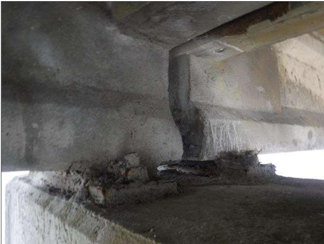
Span 172 Beam 1: 12" X 12" PATCHED AREA ON SOUTH FACE AT BENT 172.
