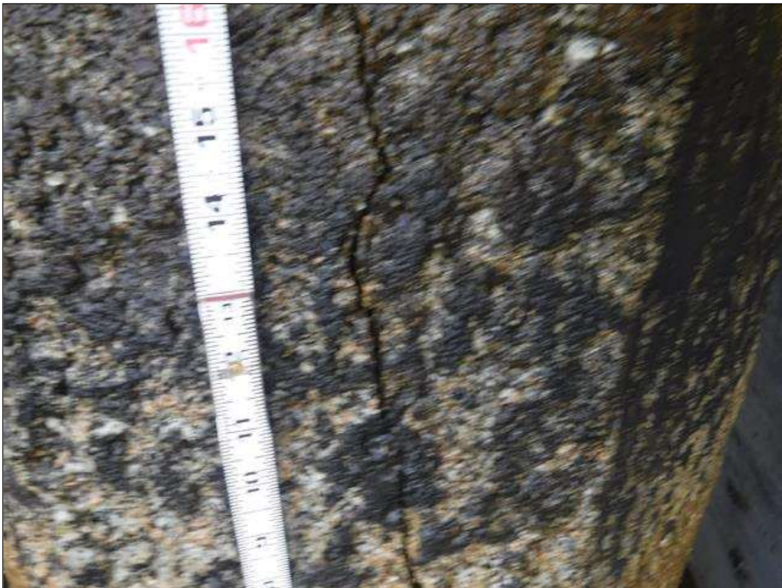
Bent 183 Pile 1: (PAR) HAIRLINE TO 1/8" CRACKS, 8' BELOW CAP, DOWN 4', MULTIPLE FACES. SCALING TO 1" DEEP WITH LOOSE AGGREGATE FROM WATERLINE TO MUDLINE.
