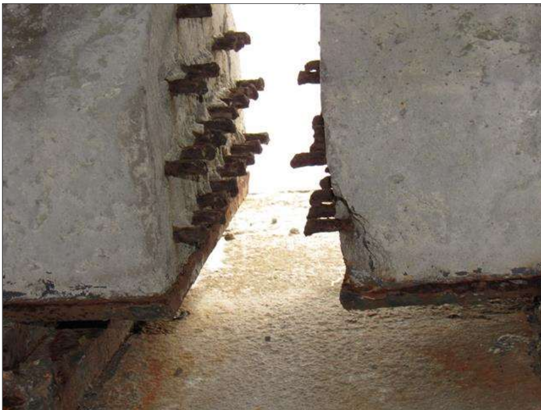
Span 68 Beam 4: 3" HIGH X 1" WIDE CORNER SPALL AT BENT 68
