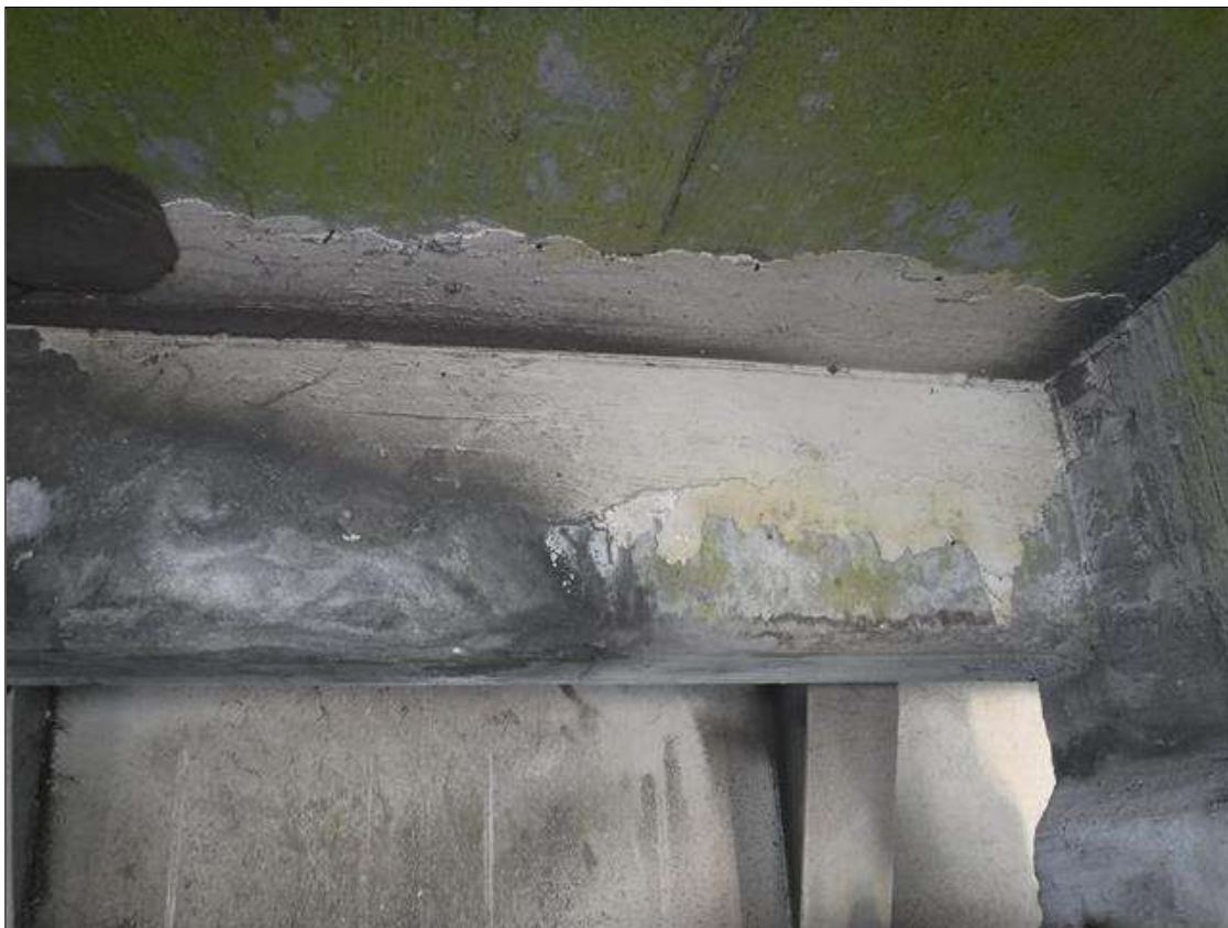
Span 118 Deck: 6' X 1' PATCHED AREAS IN EACH BAY AT BENT 117
