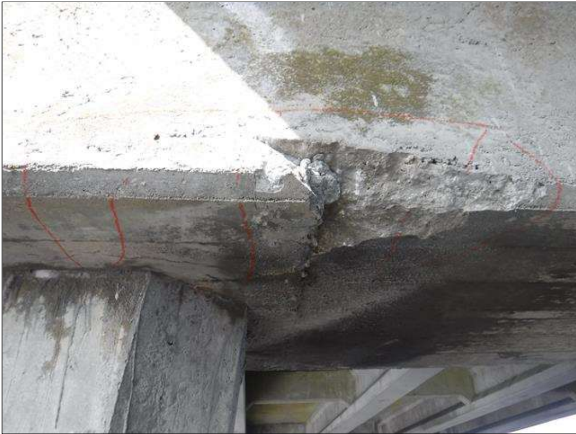
Bent 223 Cap 1: 2' X 6" X 16" DEEP DELAMINATION WITH UP TO 3" DEEP SPALL ON BOTTOM OF EAST FACE AT PILE 6
