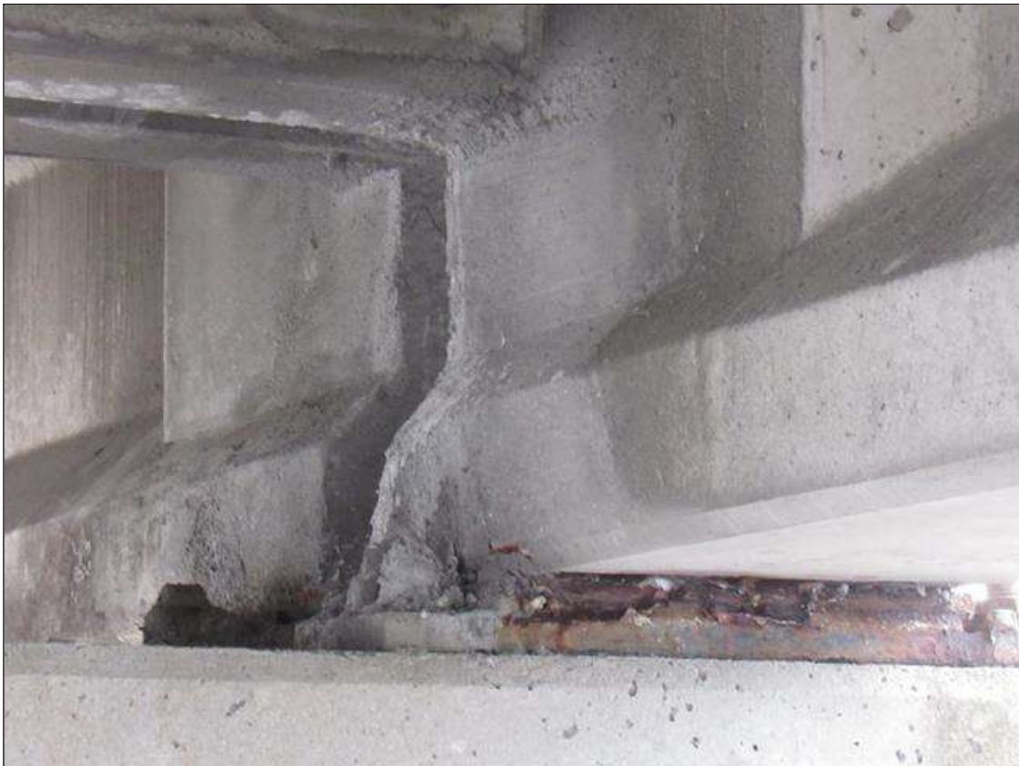
Span 33 Beam 4: 10" X 1' PATCHED AREA, NORTH FACE, AT BENT 33.
