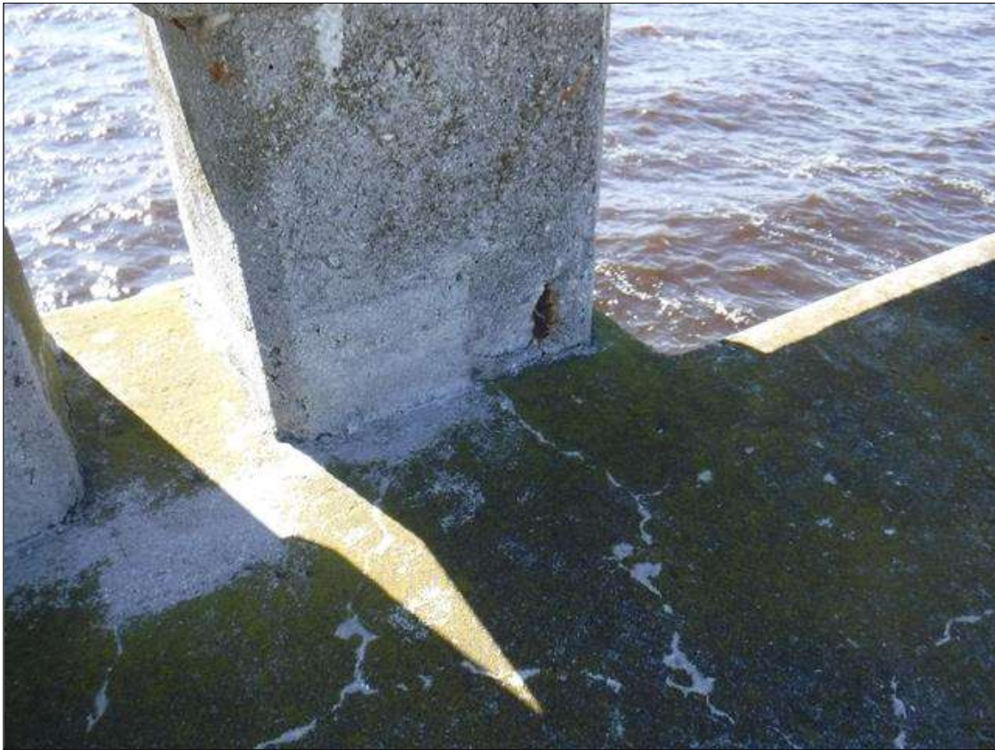
Span 84 Right Bridge Rail: 2" X 2" X 3/4" SPALL WITH EXPOSED REBAR AT BOTTOM LEFT CORNER LOCATED ON POST 6
