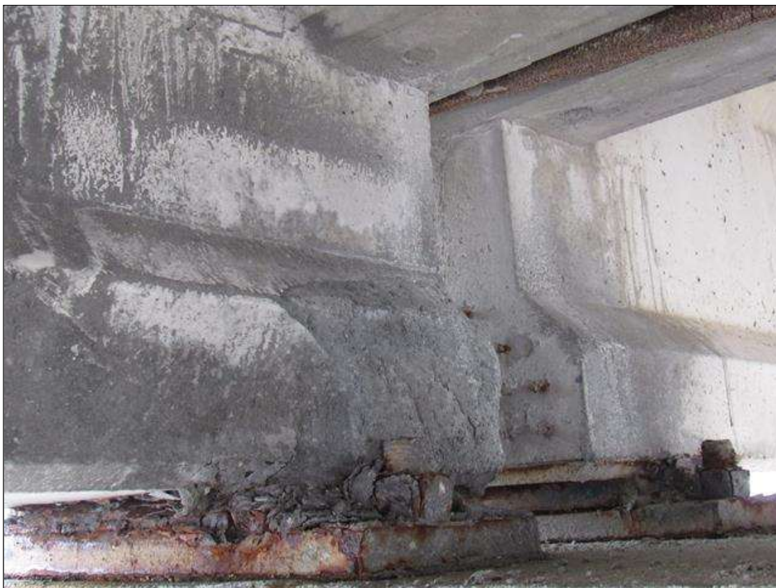
Span 48 Beam 1: 12" X 8" PATCHED AREA, NORTH FACE, 4' FROM BENT 48.
