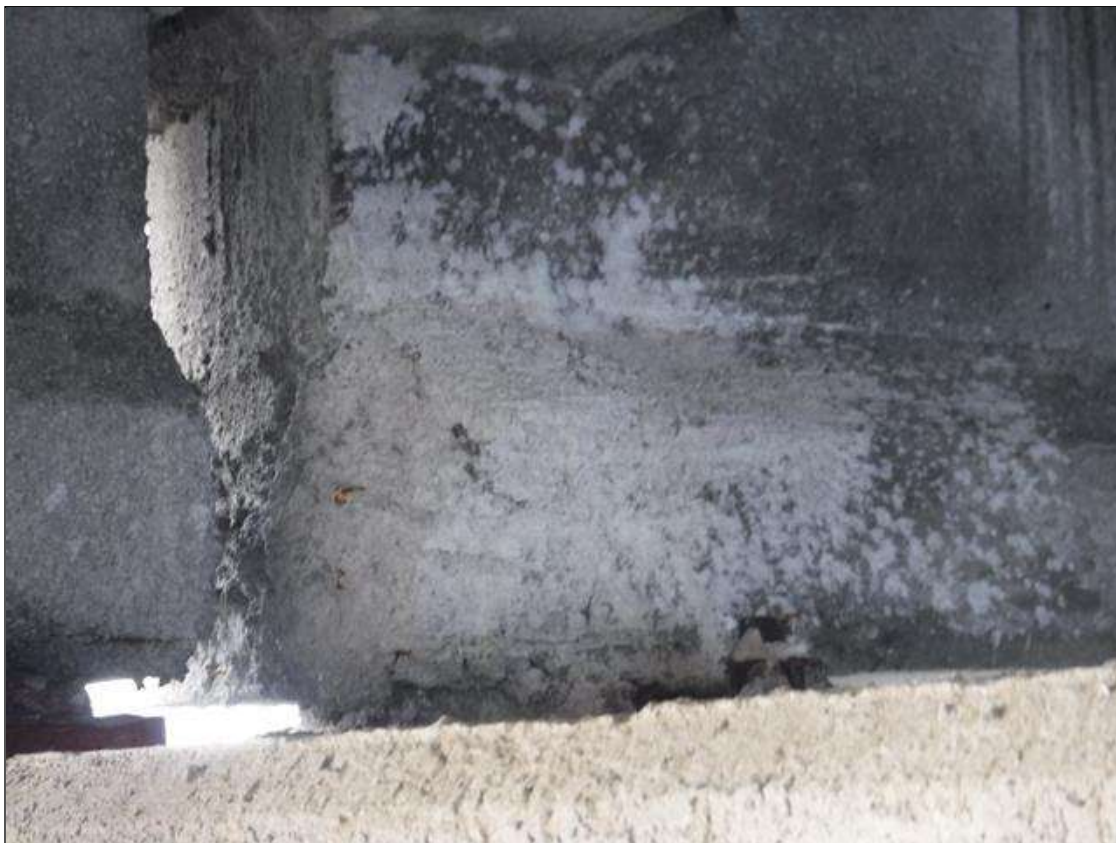
Span 153 Beam 4: 12" X 12" PATCHED AREA ON NORTH FACE AT BENT 153
