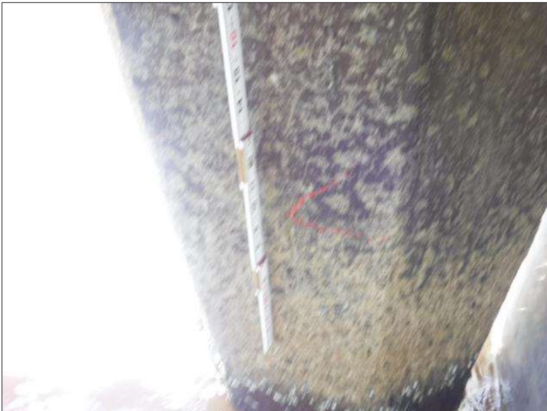
Bent 223 Pile 6: (PAR) HAIRLINE TO 1/8" CRACKS, 8' BELOW CAP, DOWN 4', MULTIPLE FACES. SCALING TO 1" DEEP WITH LOOSE AGGREGATE FROM WATERLINE TO MUDLINE.
