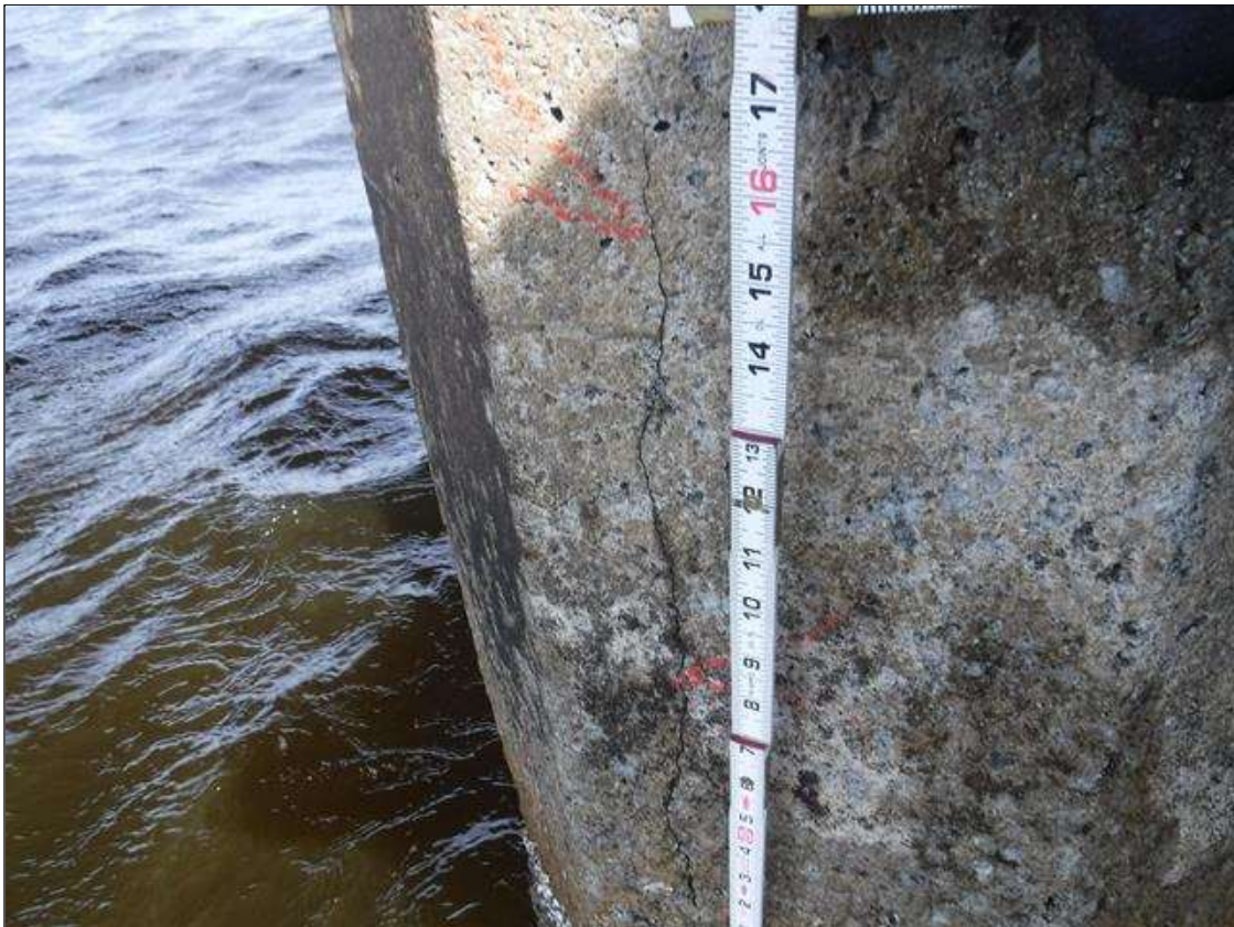
Bent 165 Pile 3: (PAR) HAIRLINE TO 1/8" CRACKS, 6' BELOW CAP, DOWN 10', MULTIPLE FACES. SCALING TO 1' DEEP WITH LOOSE AGGREGATE FROM WATERLINE TO MUDLINE.
