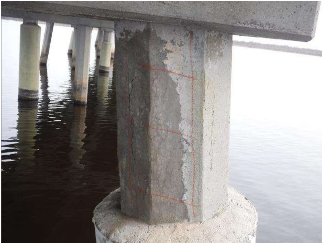
Bent 233 Pile 4: (PAR) 36" X 36" FAILED PATCHED AREA WITH UP TO 1/8" WIDE VERTICAL CRACK, WEST AND NORTH FACE, BEGINNING FROM BOTTOM OF CAP.
