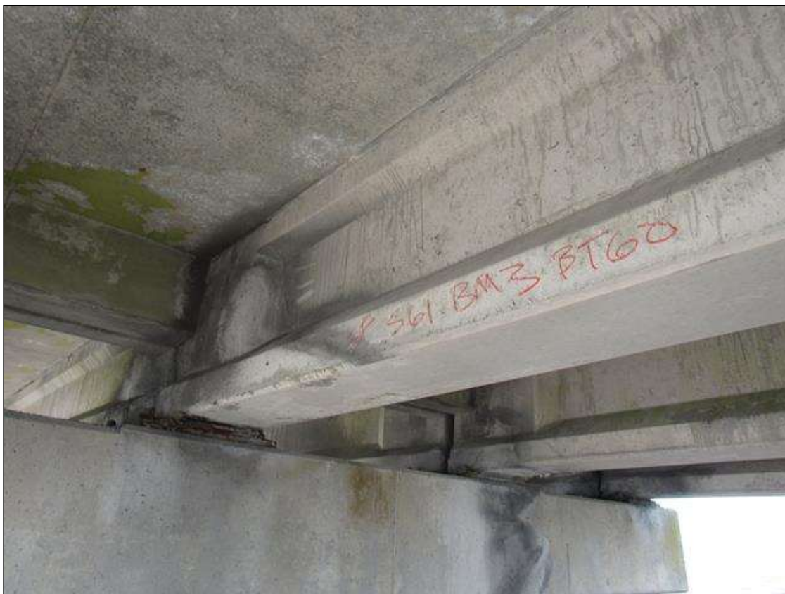
Span 61 Beam 3: 12" X 18" PATCHED AREA, SOUTH FACE, 2' FROM BENT 60.
