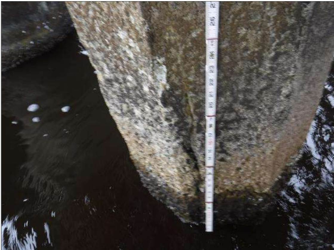
Bent 255 Pile 2: (PAR) 4' X 1/4" TO 1/2" CRACK ON NORTH FACE, 8' BELOW CAP, DOWN 4'. SCALING TO 1" DEEP WITH LOOSE AGGREGATE FROM WATERLINE TO MUDLINE.
