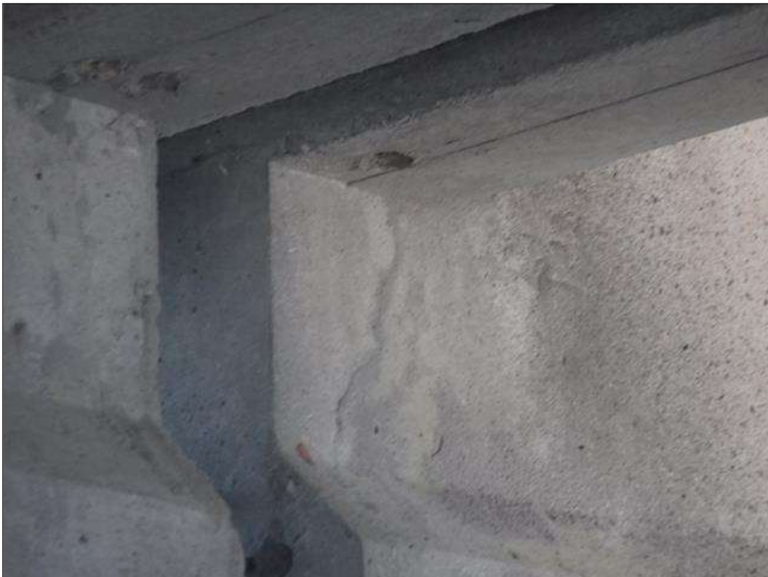
Span 25 Beam 1: 1' TALL HAIRLINE CRACK IN WEB ON SOUTH FACE AT BENT 24.
