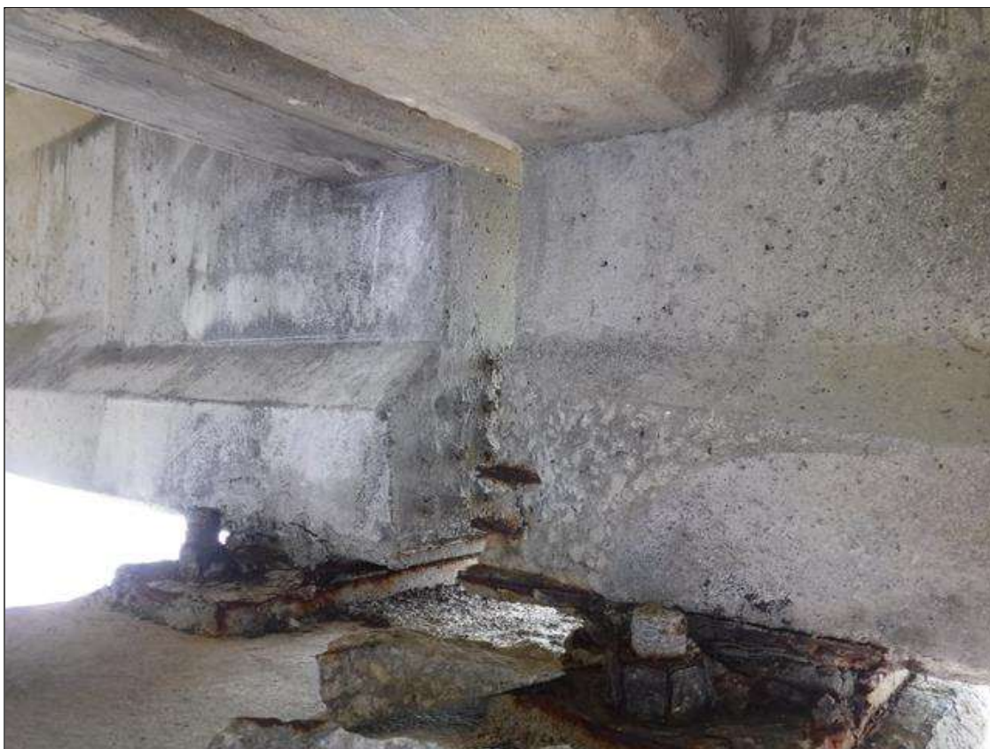
Span 147 Beam 4: (PAR) 6" X 6" X 2" DEEP SPALL WITH EXPOSED STRAND ON NORTH FACE AT BENT 147
