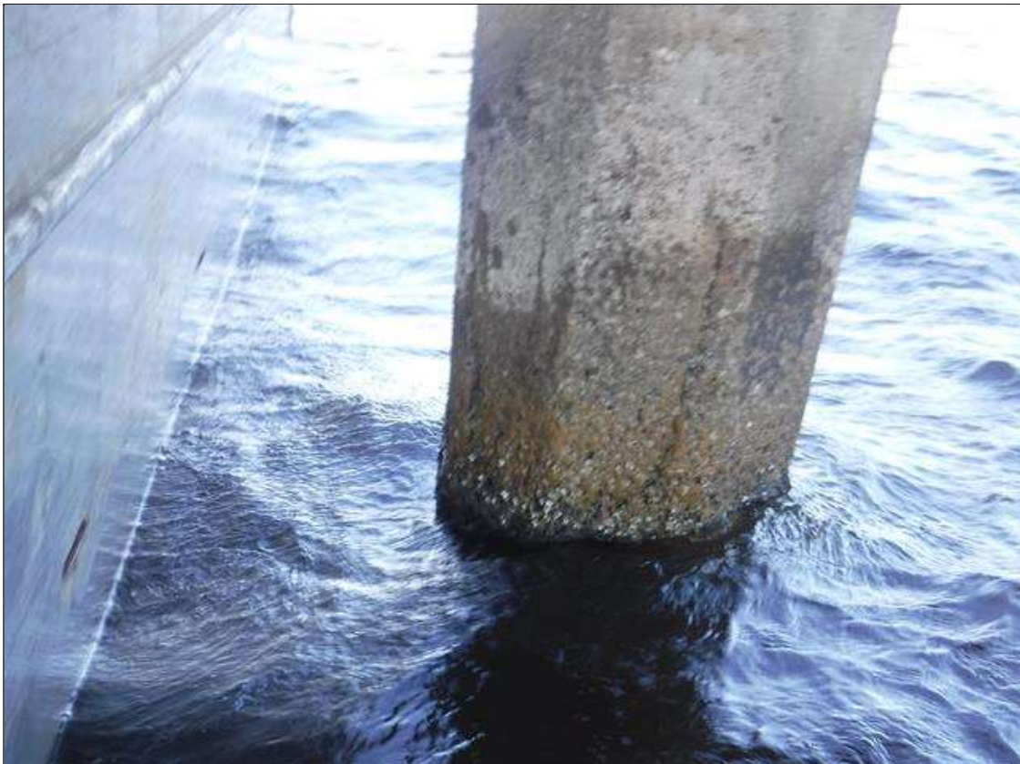
Bent 26 Saved Pile 1: (PAR) HAIRLINE TO 1/8" CRACK, 8' BELOW CAP, DOWN 6', SOUTH QUAD. SCALING TO 1" DEEP FROM WATERLINE TO MUDLINE.
