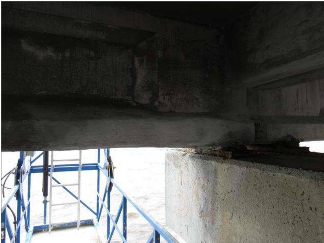
Span 51 Beam 4: 54" X 12" X 12" CORNER PATCHED AREA, NORTH FACE, AT BENT 50.
