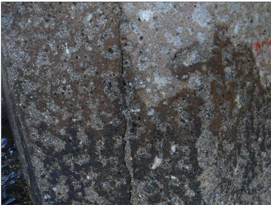
Bent 162 Pile 4: (PAR) 2' X UP TO 0.04" VERTICAL CRACK, SOUTH FACE, 9' FROM BOTTOM OF CAP, WITH ADJACENT 1' X 2' DELAMINATION.
