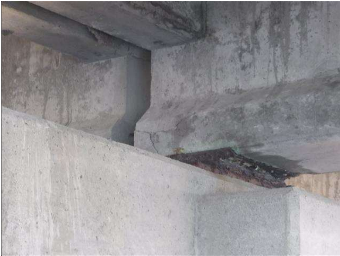
Span 17 Beam 3: 12" X 12" FAILED PATCHED AREA, NORTH FACE, AT BENT 17.
