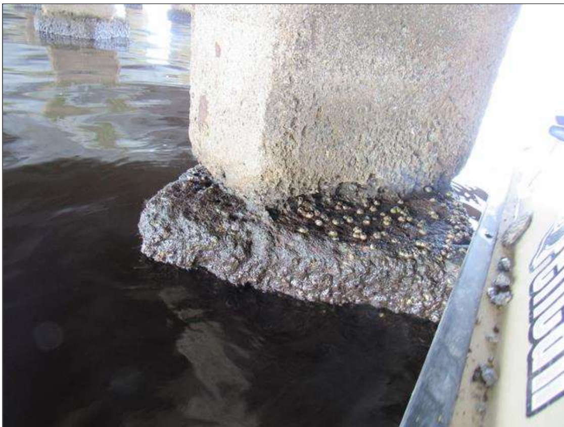
Bent 285 Pile 2: FULL PERIMETER OF PILE X 2" DEEP SPALL WITH EXPOSED REINFORCING ON EAST AND RIGHT FACE
