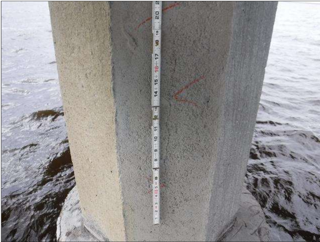
Bent 190 Pile 3: UP TO 5' X 0.009" VERTICAL CRACK ON EAST FACE
