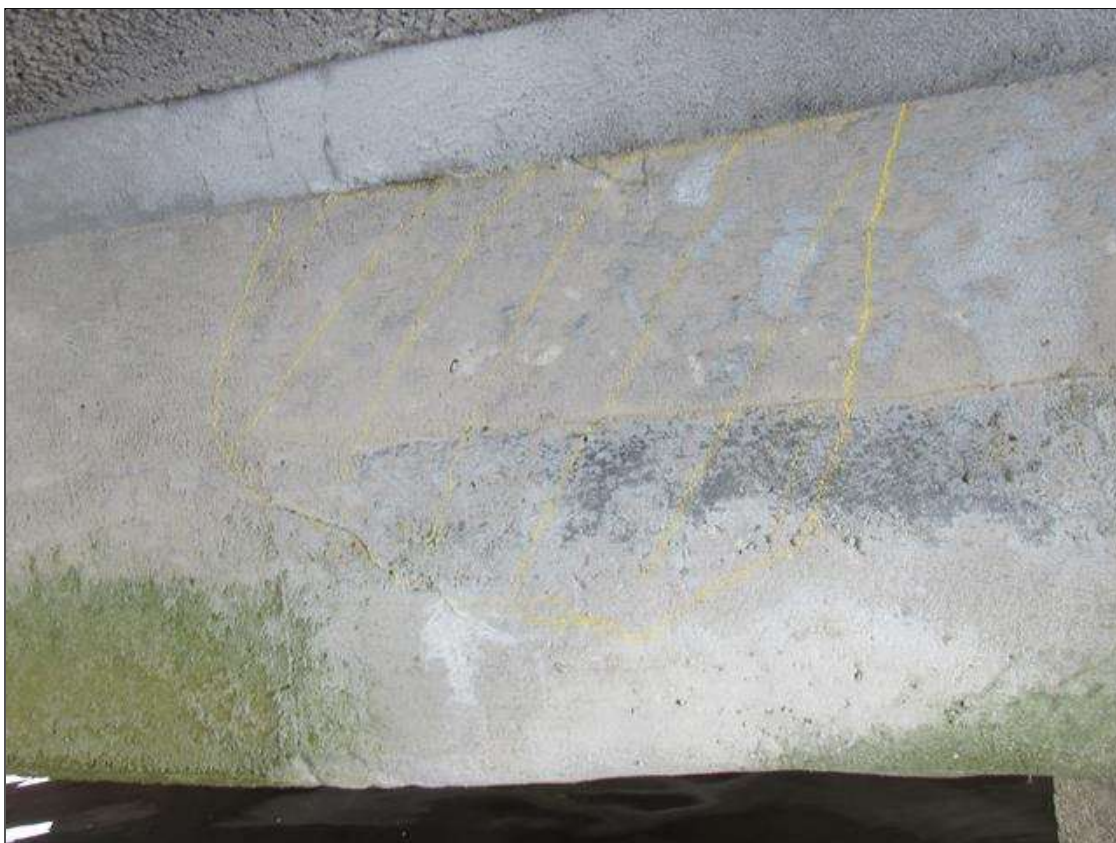
Bent 283 Cap 1: 3' X 1.5' DELAMINATION, WEST FACE, BAY 2.
