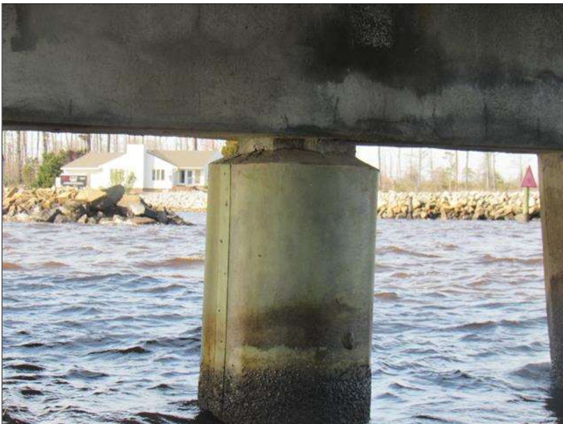
Bent 7 Saved Pile 2: PILE REPAIRED WITH 3' DIAMETER CONCRETE JACKET
