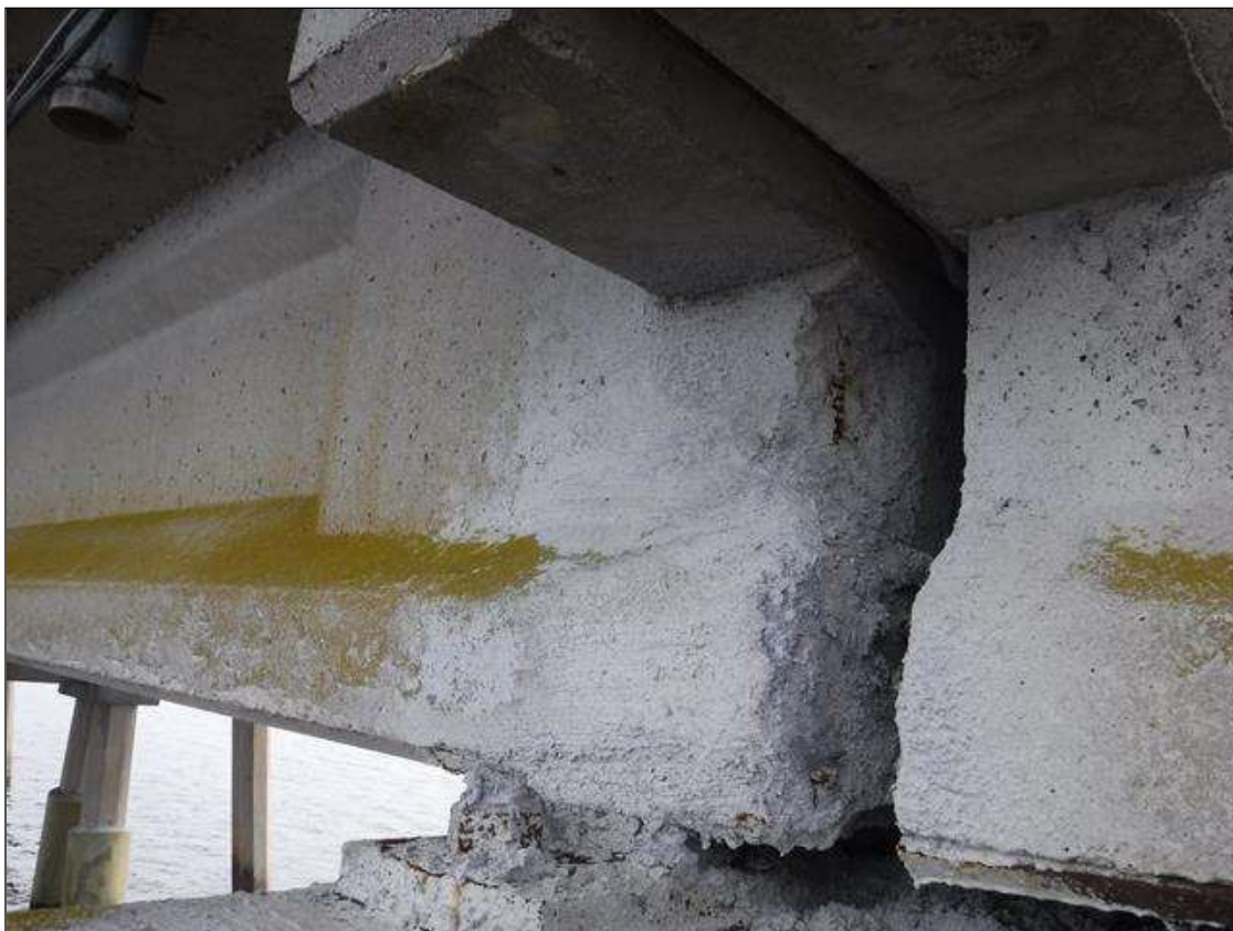
Span 101 Beam 1: 1' X 1' PATCHED AREA WITH EXPOSED REBAR, NORTH FACE, AT BENT 100.
