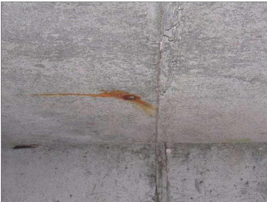
Span 65 Deck: 2" X 2" AREA OF RUST STAINING, UNDERSIDE OF DECK FACE, BETWEEN BEAMS 3 AND 4, 3' FROM BENT 64.
