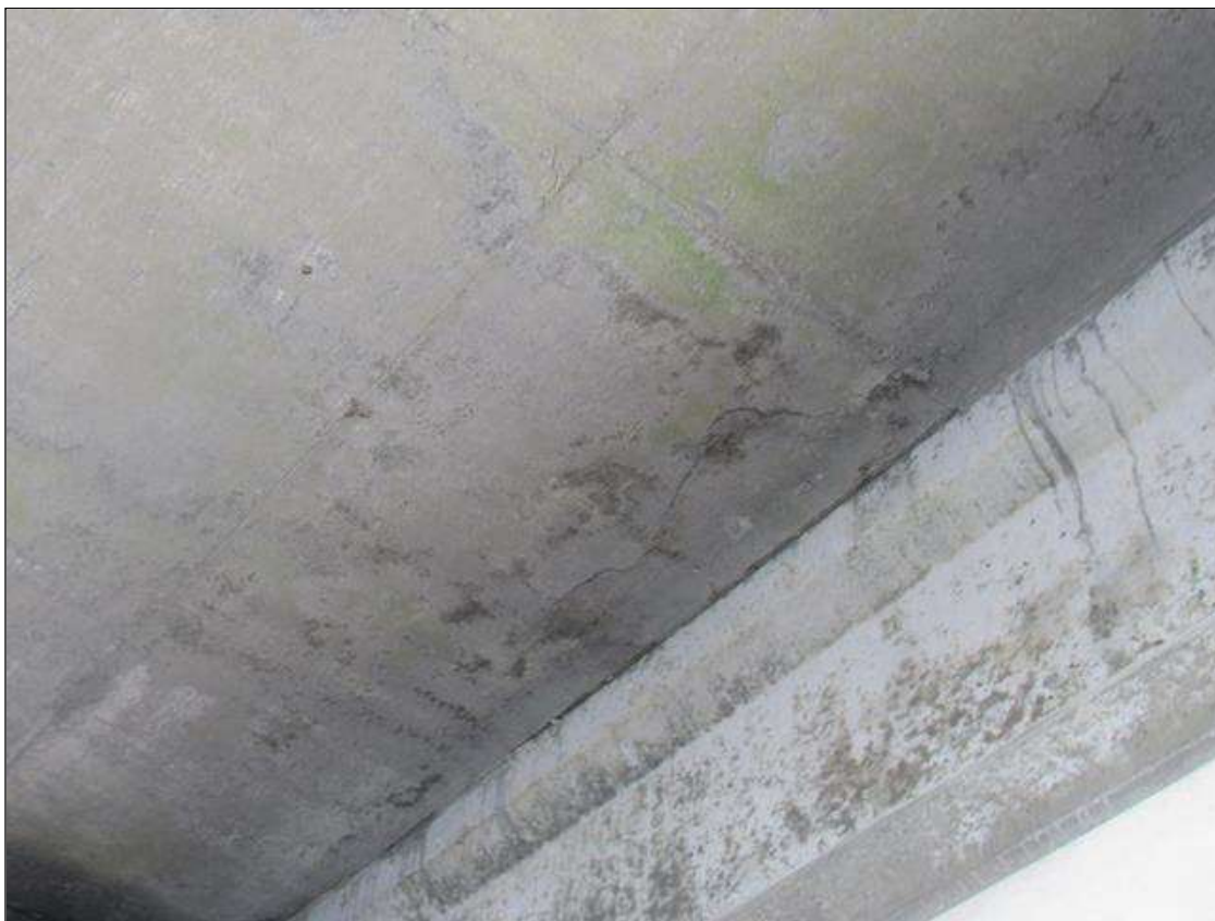
Span 269 Deck: 4' X UP TO 18" DELAMINATION ON UNDERSIDE OF DECK LOCATED LEFT OF BEAM 3, 6' FROM SPAN 270
