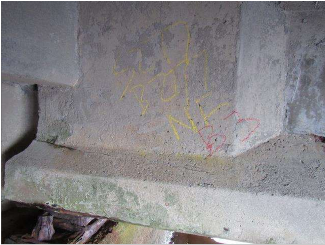
Span 277 Beam 3: UP TO 24" X 8" CRACKED DELAMINATION ON NORTH AND SOUTH FACES, AT BENT 277.
