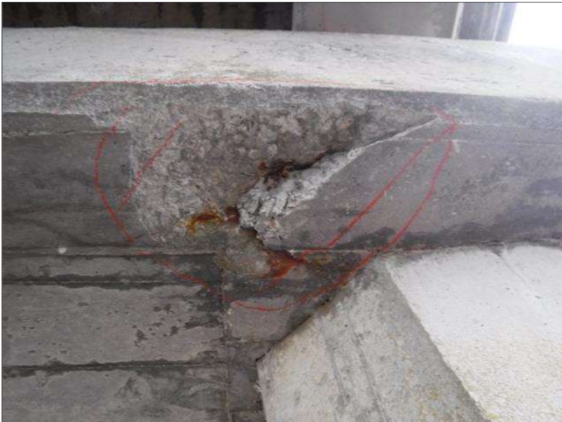
Bent 238 Cap 1: (PAR) 12" X 12" X 1.5" SPALL, WITH EXPOSED REINFORCING, WITH ADJACENT 12" X 6" DELAMINATION, BOTTOM FACE, BENEATH BEAM 1.
