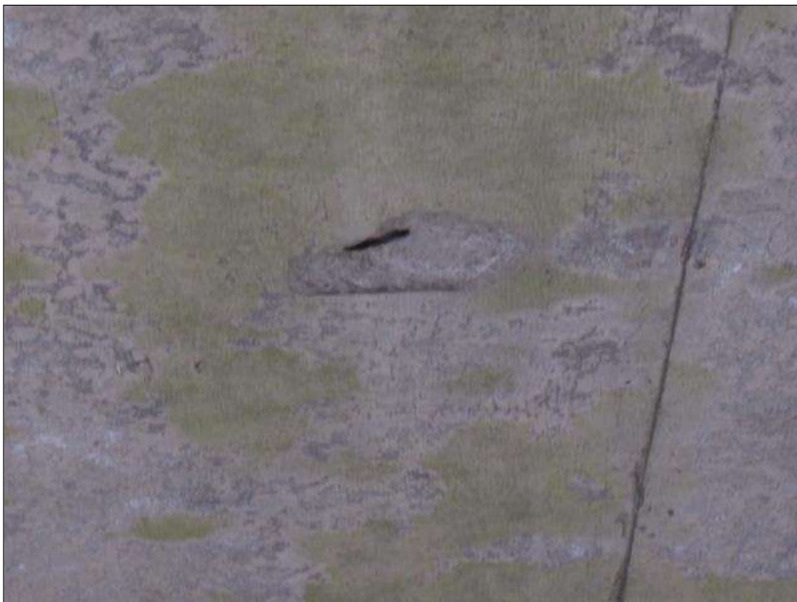
Span 31 Deck: 8" DIAMETER X 1" DEEP SPALL WITH EXPOSED REBAR ON BOTTOM FACE LOCATED ON BAY 2, 20' FROM BENT 30
