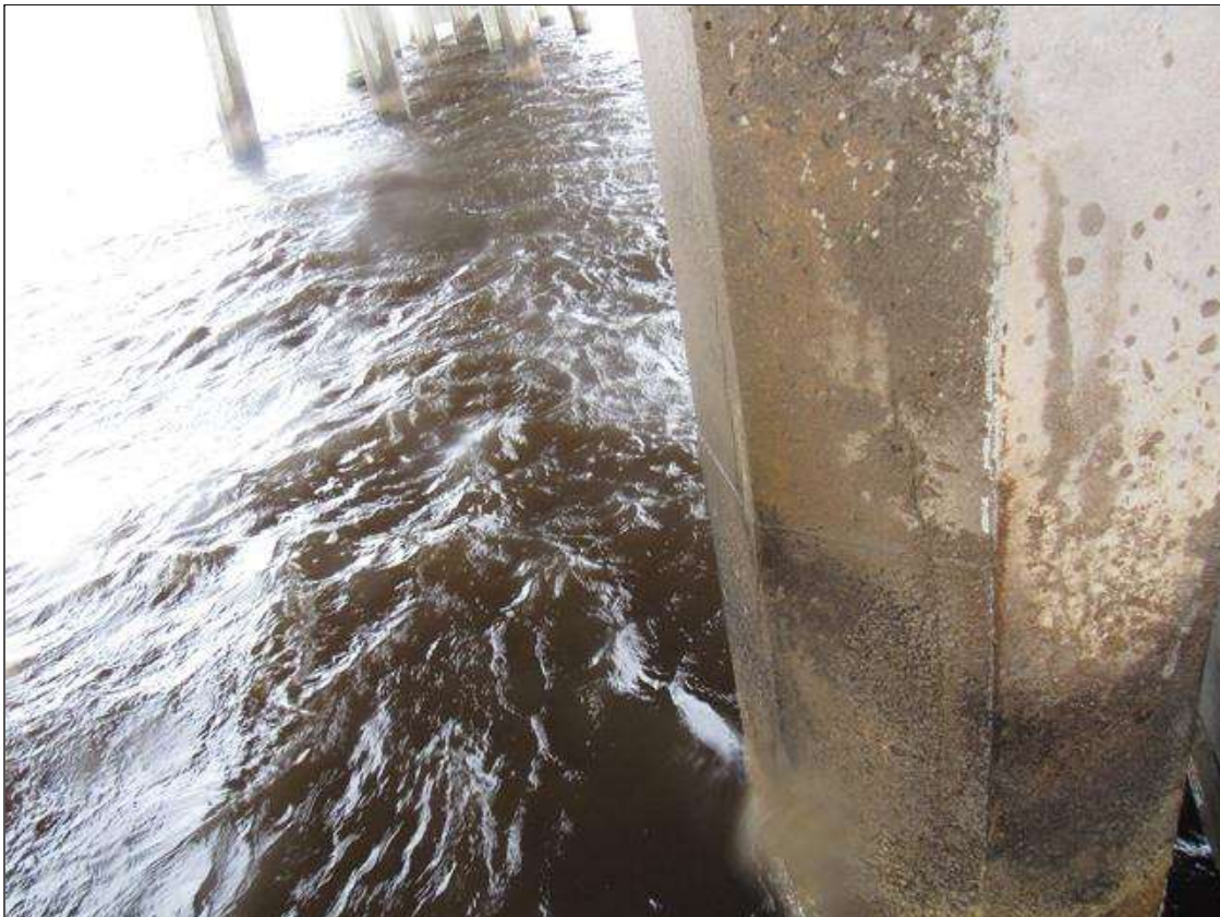
Bent 63 Pile 4: 4' X 1' DELAMINATION, NORTH FACE, 8' FROM BOTTOM OF CAP.
