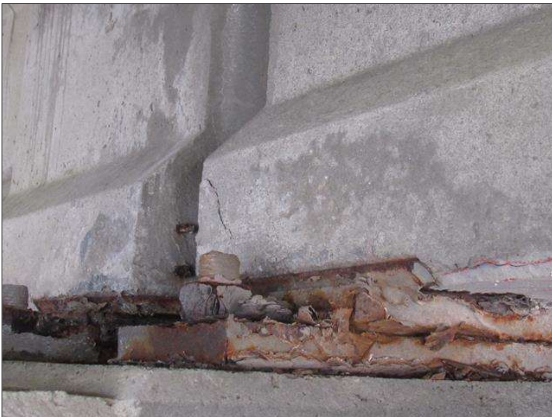
Span 34 Beam 3: 4" X 4" DELAMINATION ON SOUTH FACE AT BENT 33
