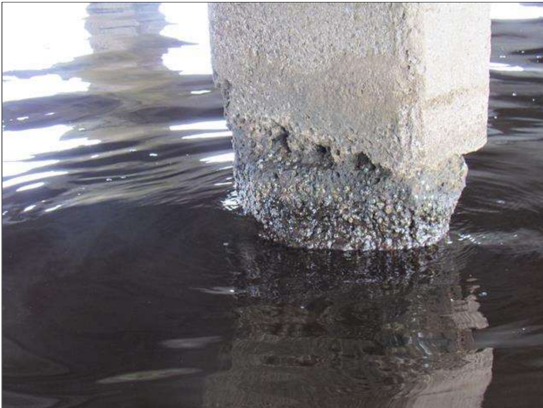
Bent 284 Pile 3: (PAR) 24" X 24" X 24" SPALL, WITH EXPOSED REBAR WITH COMPLETE SECTION LOSS, WEST FACE OF COLUMN FOOTING.
