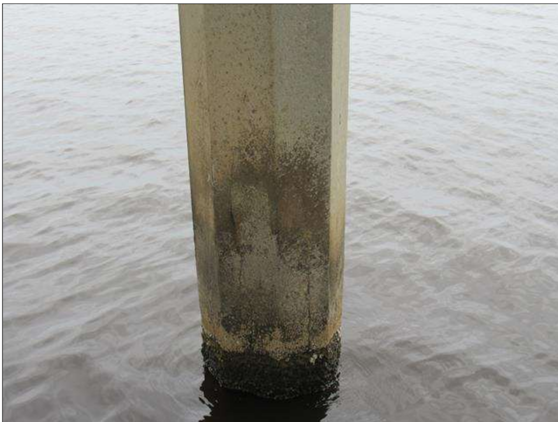
Bent 47 Saved Pile 4: 3' X 1' DELAMINATION, NORTH FACE, 7' FROM BOTTOM OF CAP.
