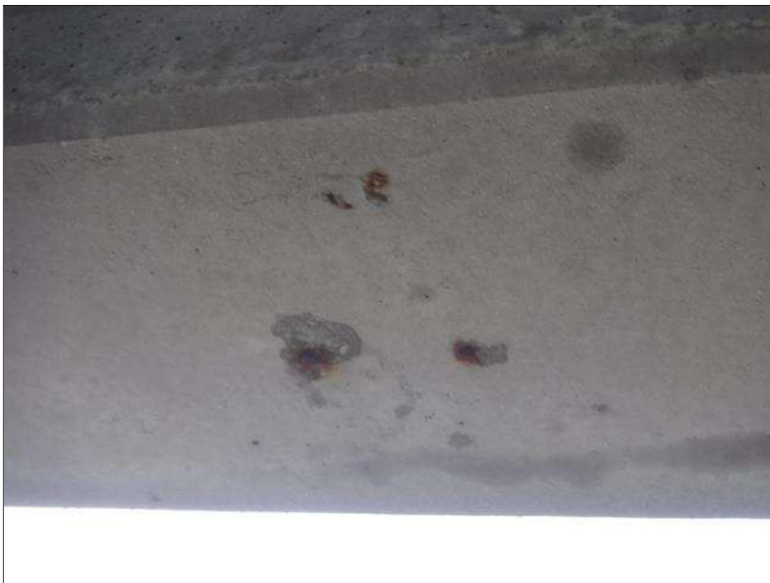
Span 151 Beam 4: (2) UP TO 3" DIAMETER X 1/2" SPALLS, WITH EXPOSED REINFORCING, BOTTOM FACE, 2' FROM BENT 150.
