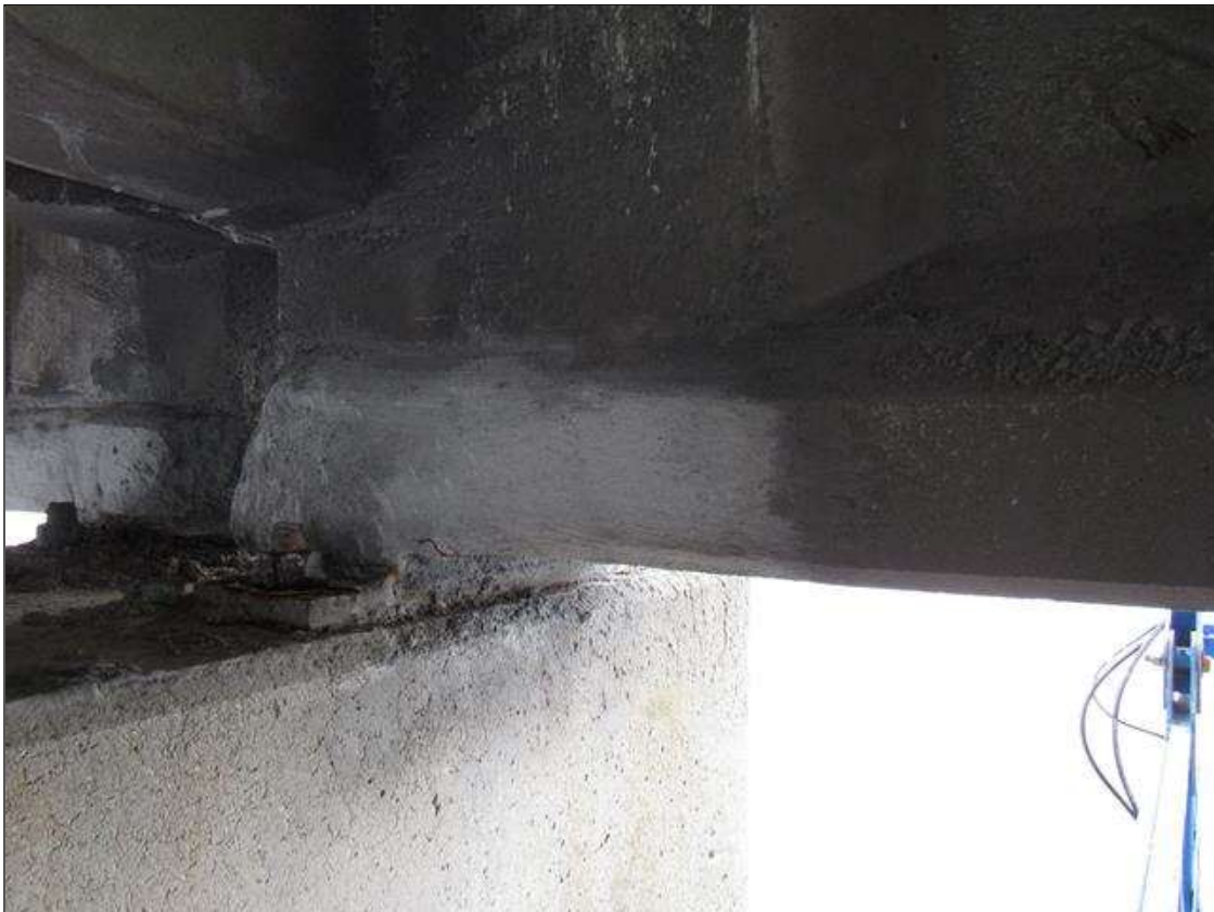
Span 59 Beam 4: 30" X 12" PATCHED AREA, NORTH FACE, AT BENT 59.
