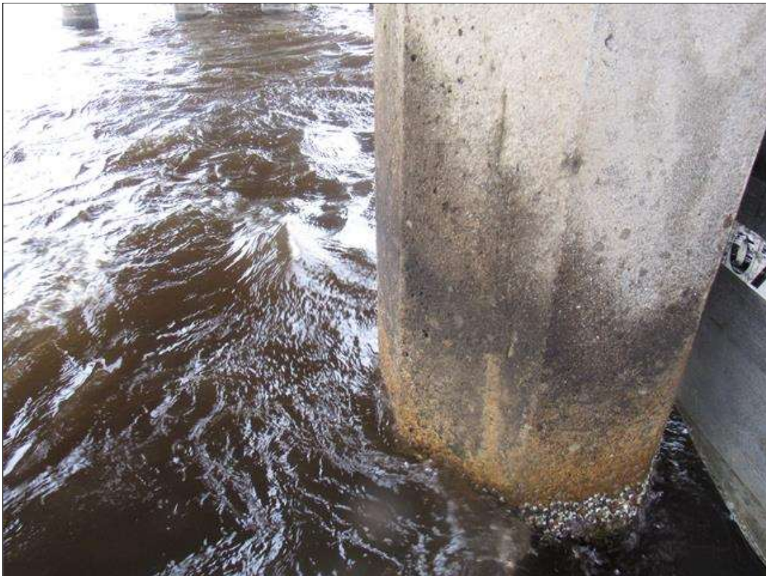
Bent 103 Pile 3: (PAR) UP TO 3' X 0.012" VERTICAL CRACKS, NORTH FACE, BEGINNING 9' FROM BOTTOM OF CAP, WITH ADJACENT 2' X UP TO 1' DELAMINATION.
