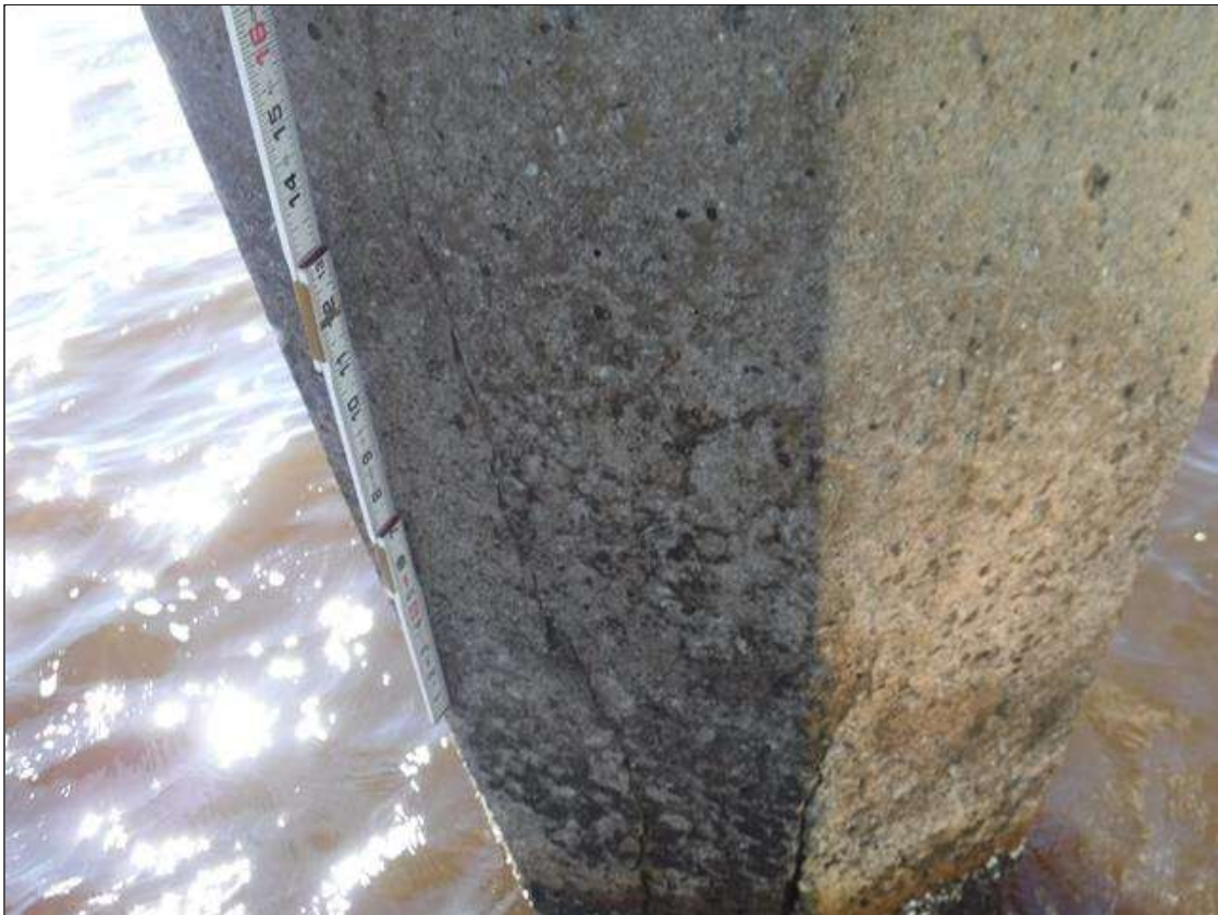
Bent 15 Saved Pile 4: (PAR) HAIRLINE TO 1/4" CRACKS, 10' BELOW CAP, DOWN 6', MULTIPLE FACES. SCALING TO 1" DEEP FROM WATERLINE TO MUDLINE.
