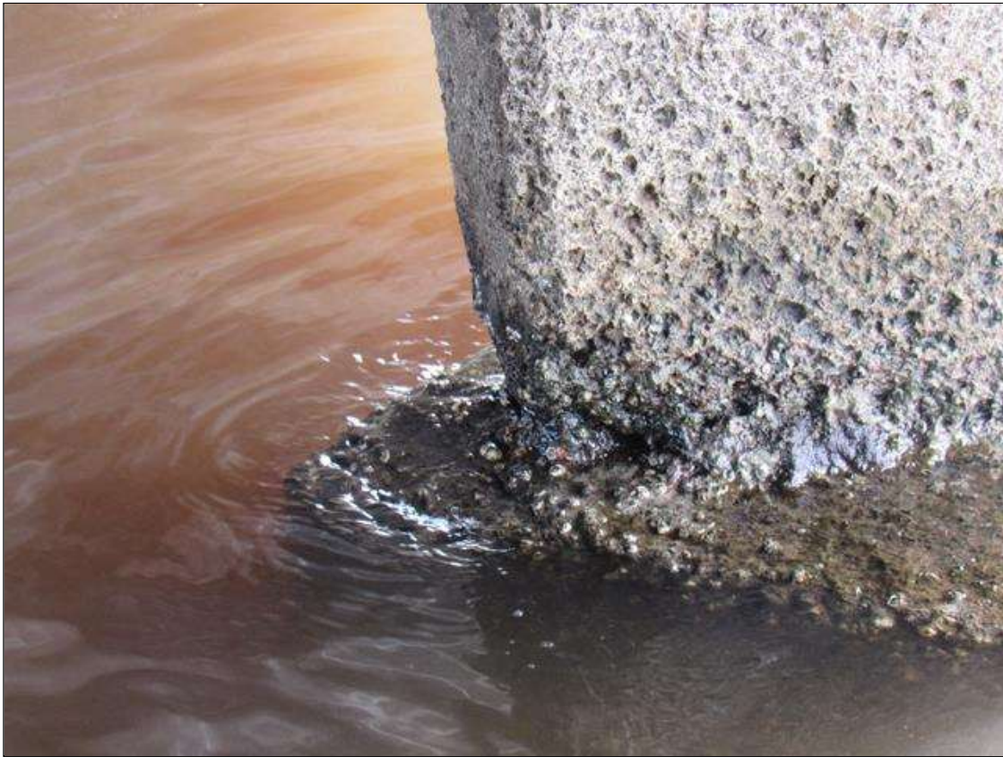
Bent 288 Pile 4: UW: SCALING AROUND BASE OF COLUMN AND TOP OF FOOTING 3" - 6" DEEP X 8" HIGH X 360*, EXPOSED REBAR WITH 25% SECTION LOSS.
