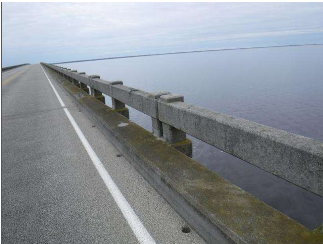
TYPICAL CONCRETE RAIL
