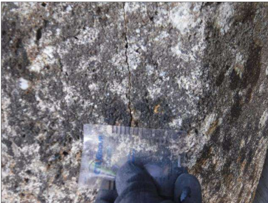
Bent 120 Saved Pile 2: (PAR) UP TO 12' X 0.03" VERTICAL CRACKS, AT RANDOM THROUGHOUT, EXTENDING BELOW WATERLINE.
