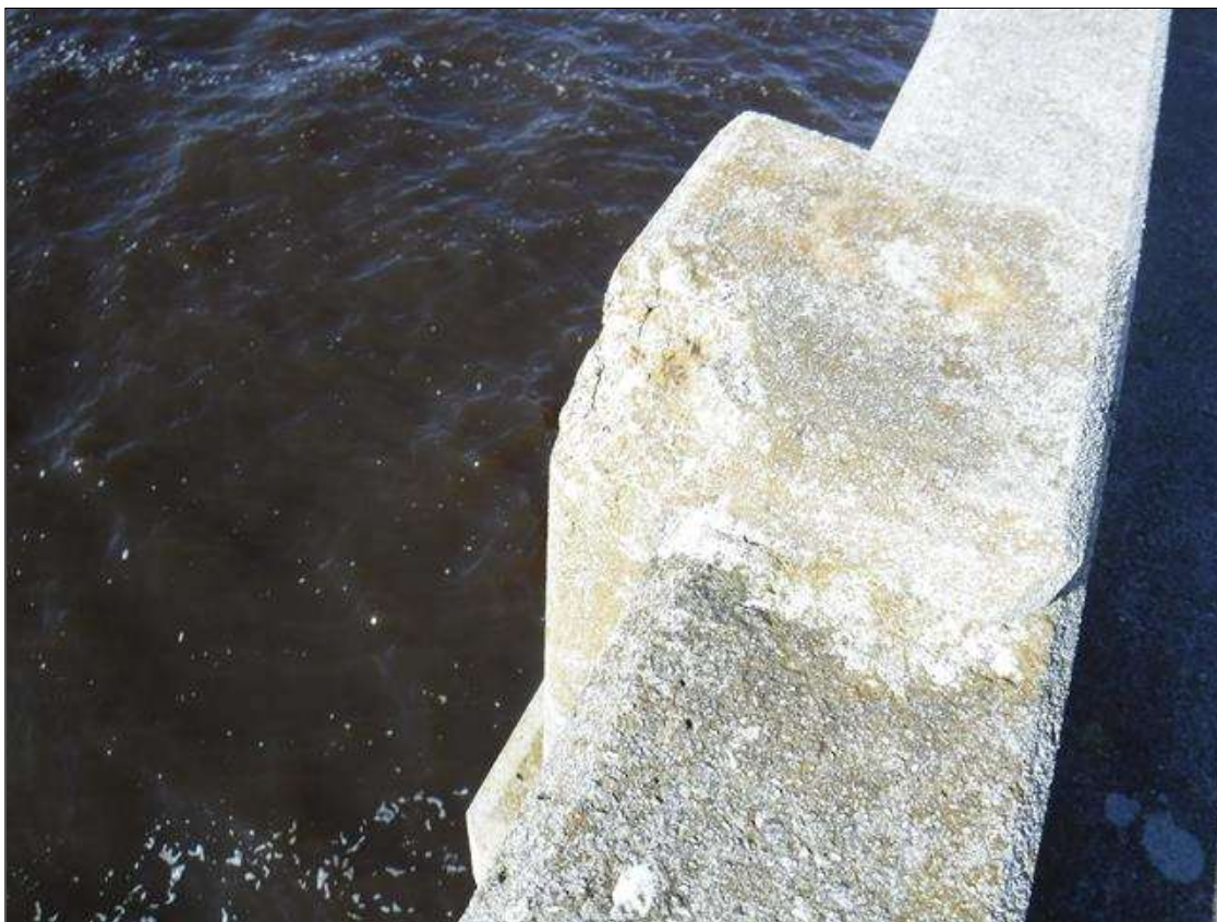
Span 15 Right Bridge Rail: (2) UP TO 6" X 4" X 3" SPALLS, WITH EXPOSED REINFORCING, AT RANDOM THROUGHOUT TOP OF RAIL POSTS.
