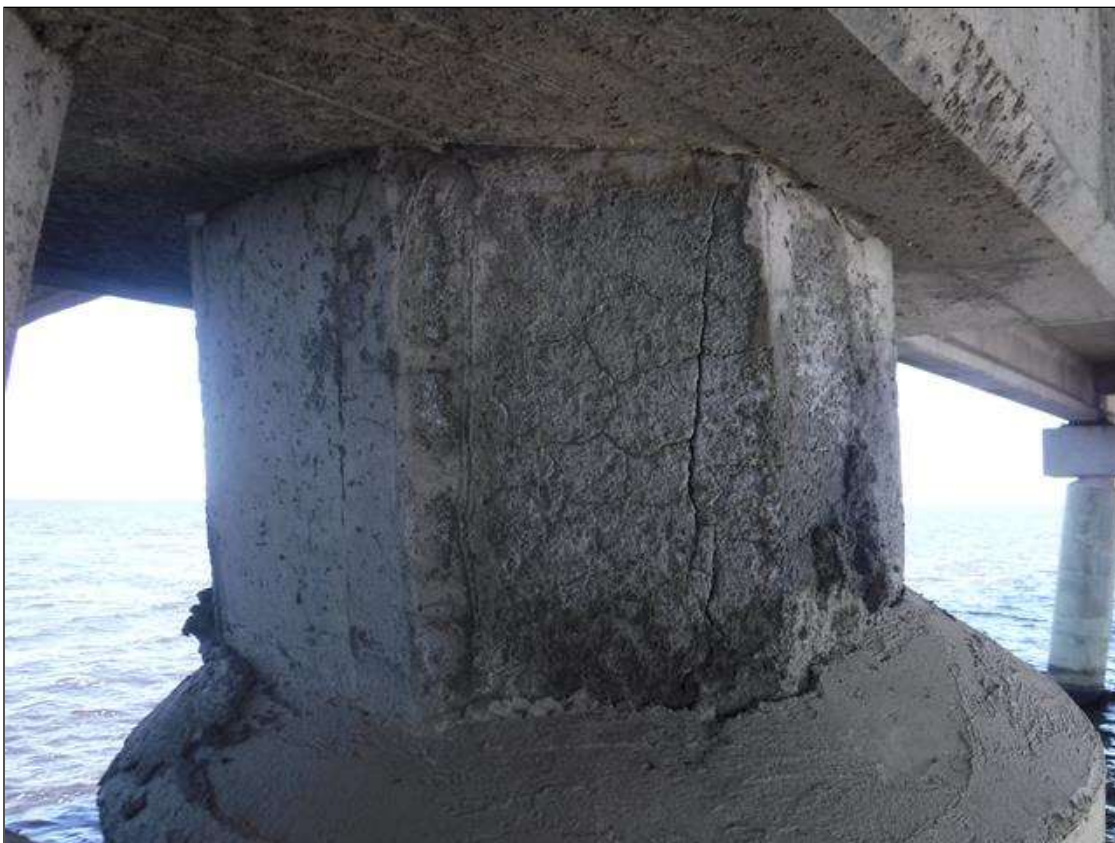
Bent 21 Saved Pile 3: 2' X 1' WIDE DELAMINATION ON SOUTHWEST FACE BELOW CAP
