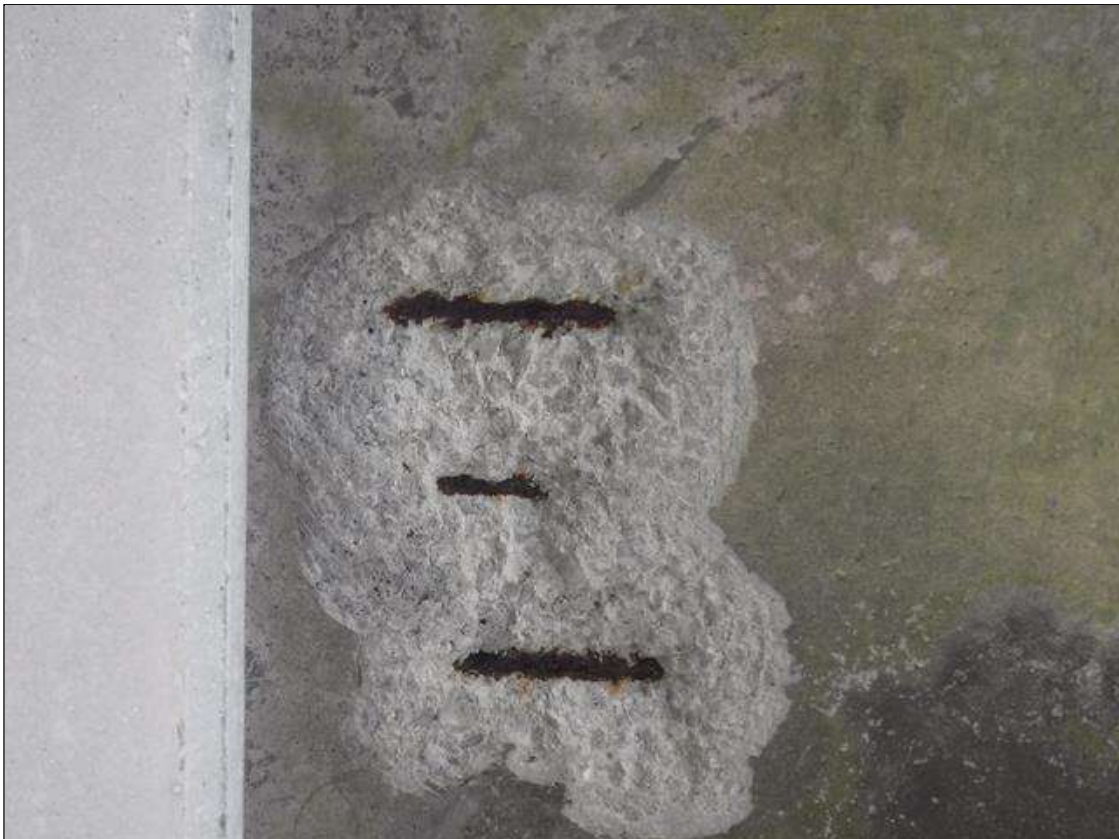
Span 236 Deck: (PAR) 2' DIAMETER X 1" DEEP SPALL WITH EXPOSED REINFORCEMENT IN DECK UNDERSIDE BAY 2, 5' FROM BENT 235
