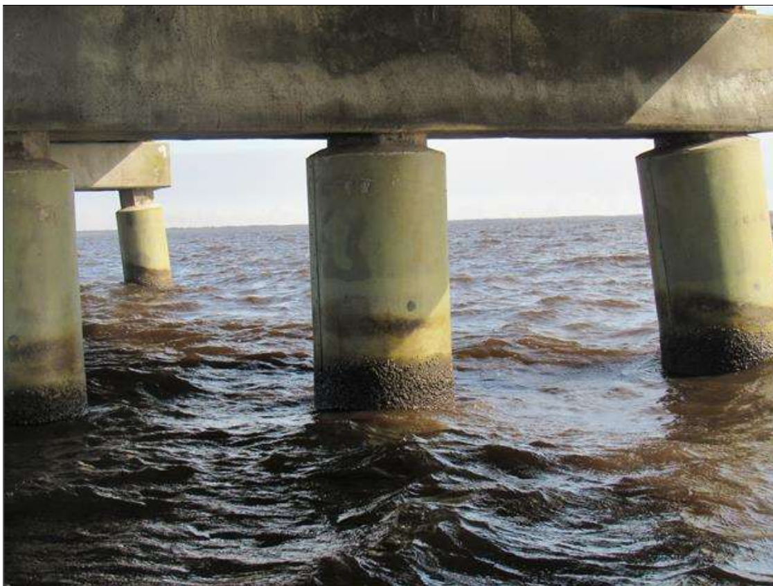
Bent 8 Saved Pile 3: PILE REPAIRED WITH 3' DIAMETER CONCRETE JACKET, OTHER PILES SIMILAR
