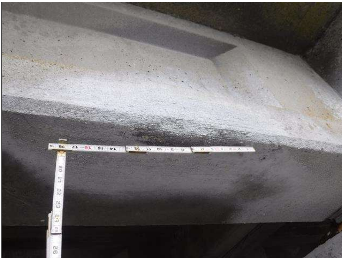
Span 236 Beam 1: 24" LONG X 6" TALL PATCHED AREA ON BOTTOM FACE 5' FROM BENT 235.
