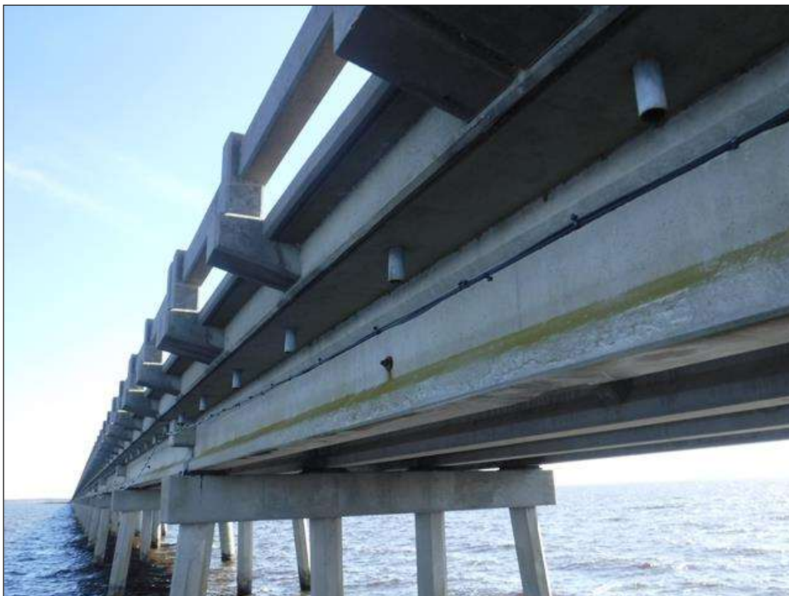
UTILITY ALONG NORTH OVERHANG, SPAN 6 SHOWN
