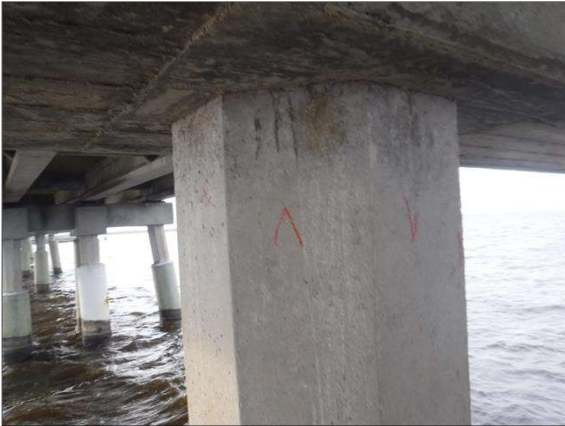
Bent 136 Saved Pile 3: 32" LONG X 0.006" HORIZONTAL CRACK ON EAST FACE 11" FROM TOP
