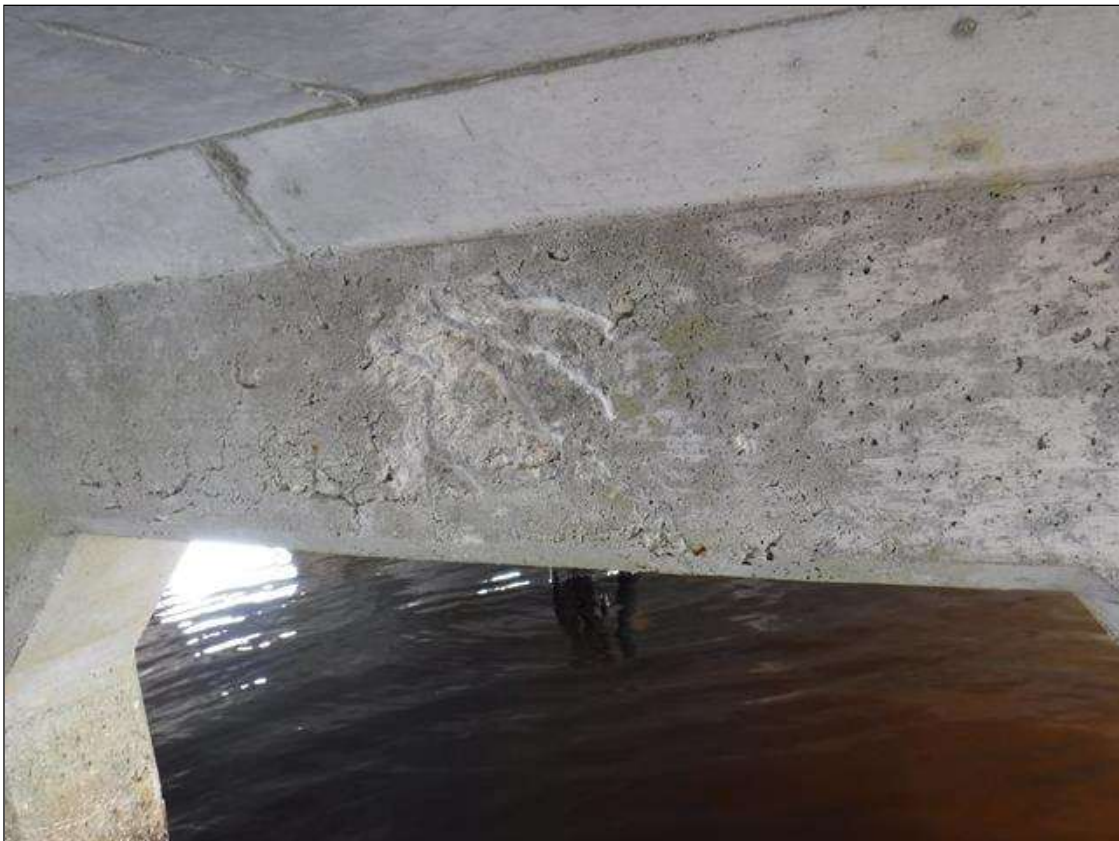
Bent 303 Cap 1: 8" X 6" X 2" SPALL, EAST FACE, BAY 1.
