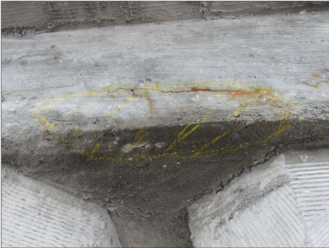
Bent 41 Cap 1: 16" X 6" DELAMINATION ON NORTH FACE LOCATED AT BOTTOM OF BLOCK-OUT BETWEEN PILES 2 AND 3, NORTH EDGE, DELAMINATION HAS RUST STAINING
