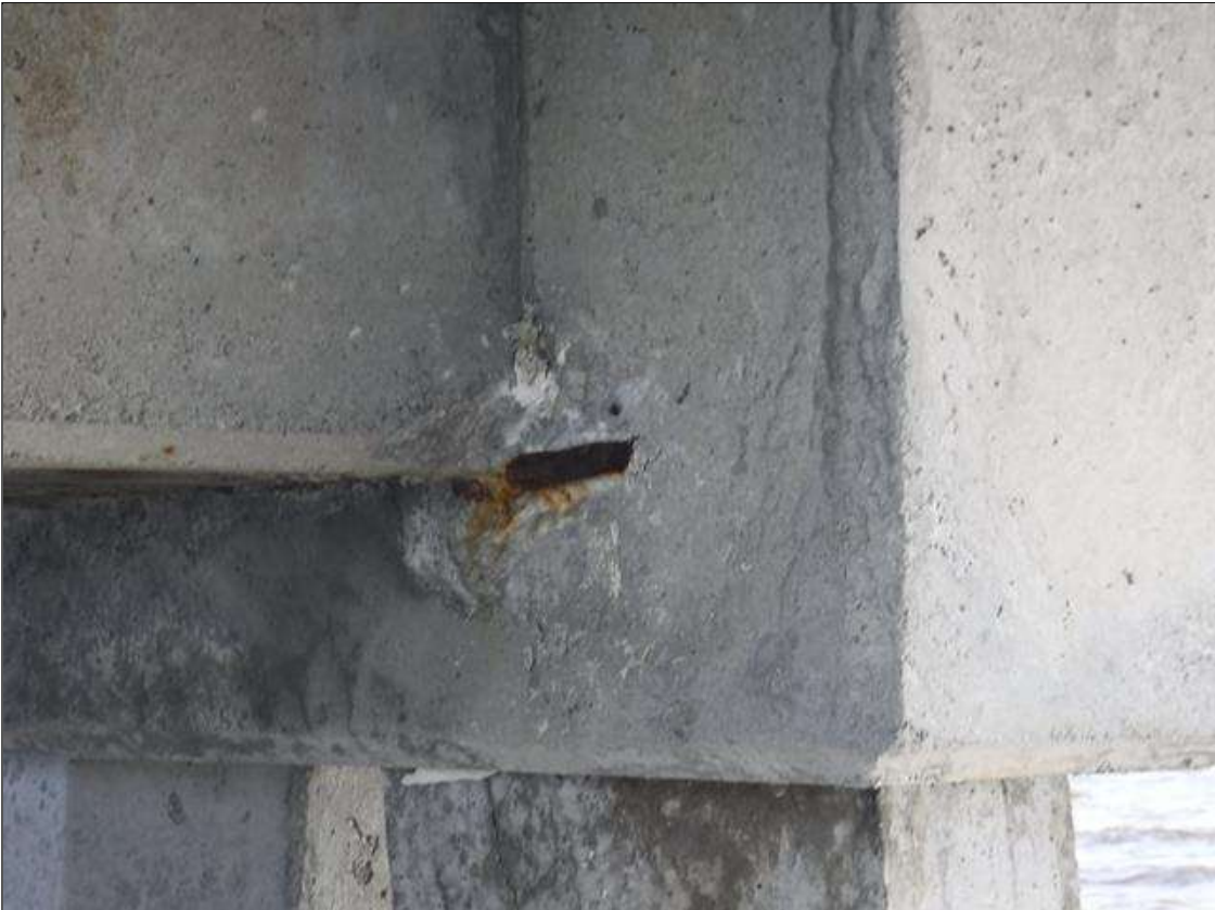
Bent 127 Cap 1: (PAR) 10" X 6" X 2" SPALL, WITH EXPOSED REINFORCING, NORTH FACE OF PILE 4 AND 5 BLOCK-OUT. REINFORCING HAS 10% SECTION LOSS
