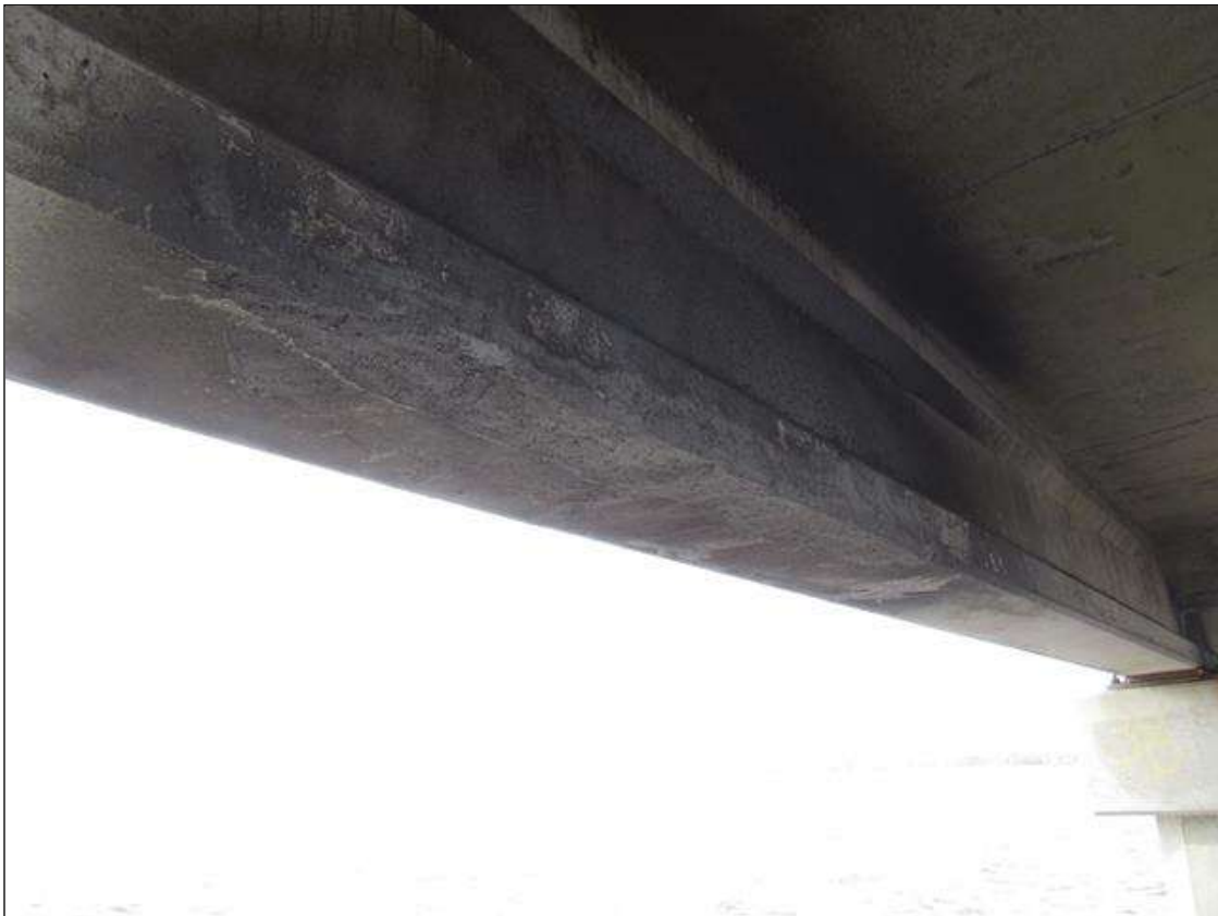
Span 39 Beam 4: 7' X UP TO 7" PATCHED AREA, BOTTOM FACE, EXTENDING 8" ONTO NORTH FACE, 18' FROM BENT 38.
