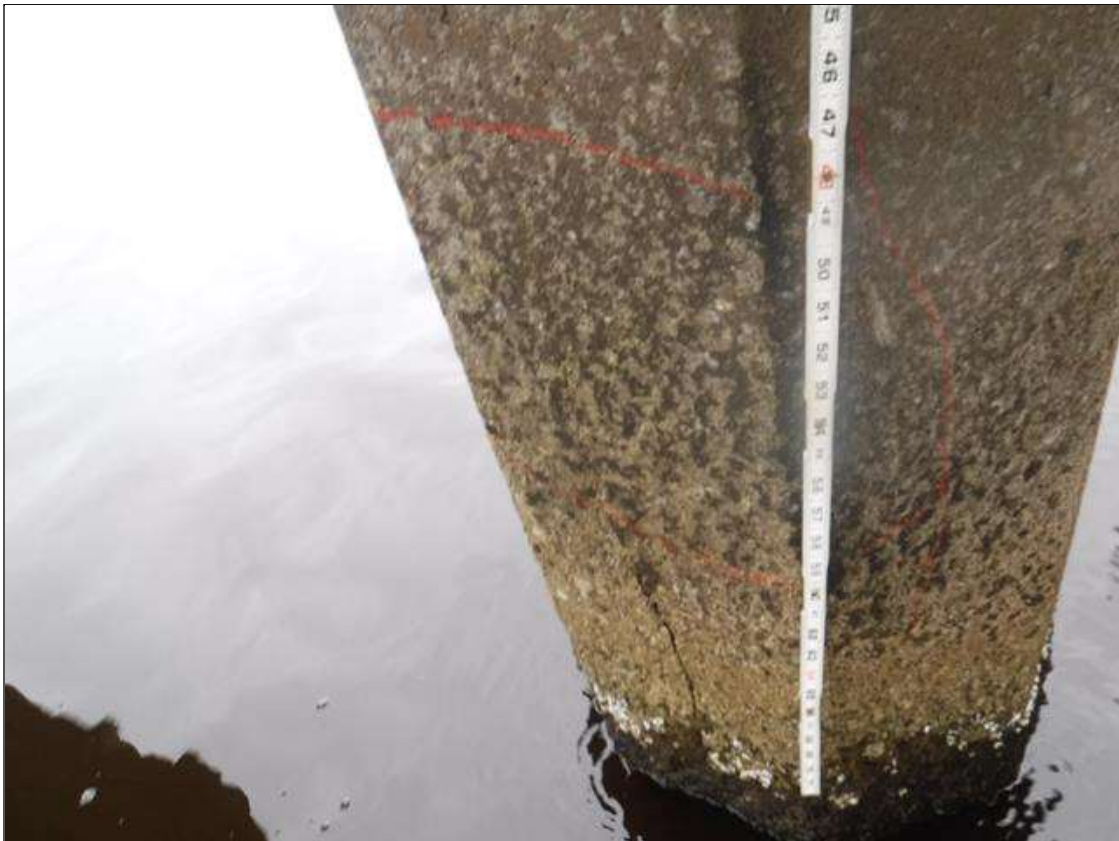
Bent 245 Pile 6: (PAR) (2) UP TO 3' X UP TO 1/8" VERTICAL CRACKS WITH 3' X 2' SURROUNDING DELAMINATION ON NORTH FACE, BEGINNING 7' FROM BOTTOM OF CAP, AT RANDOM THROUGHOUT.
