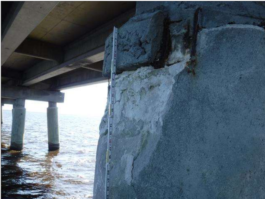
Bent 19 Saved Pile 2: (PAR) 2' X 18" X UP TO 1" DEEP SPALL WITH EXPOSED REBAR ON NORTH FACE, 2' FROM BOTTOM OF CAP. REBAR HAS COMPLETE SECTION LOSS.
