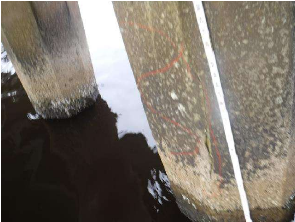
Bent 243 Pile 4: (PAR) 24" X 12" DELAMINATION, NORTH FACE, 8' FROM BOTTOM OF CAP.
