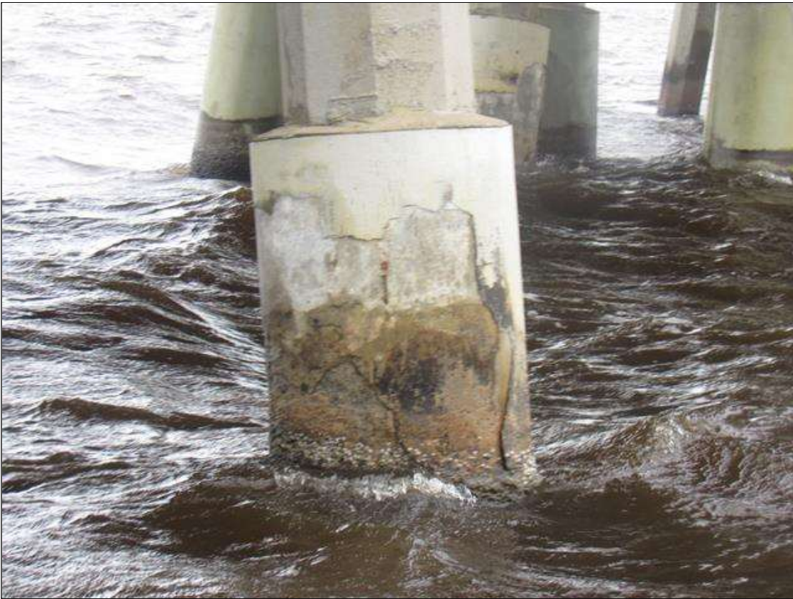
Bent 84 Pile 4: JACKETED PILE HAS EXPOSED REINFORCING, BEGINNING 7' FROM BOTTOM OF CAP AND EXTENDING BELOW WATERLINE.
