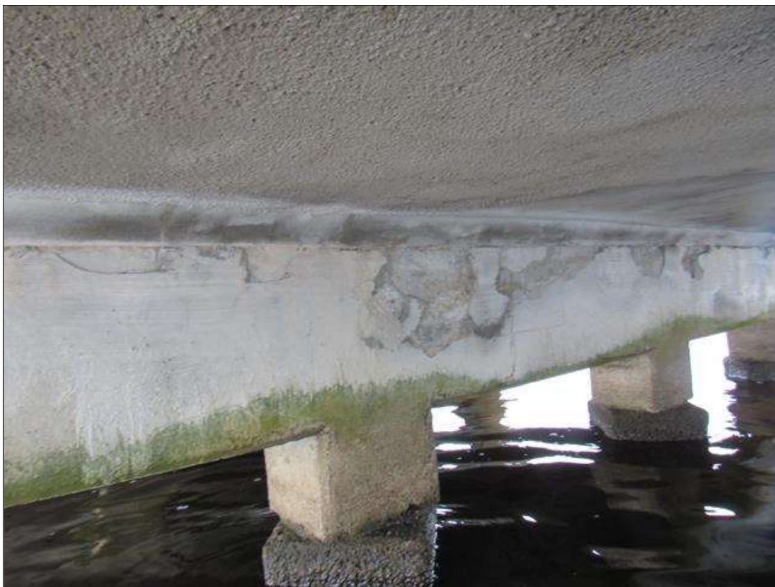
Bent 283 Cap 1: (PAR) 12' X UP TO 17" X 2" DEEP SPALL, EAST FACE, BAYS 2 AND 3. SPALL IS CAUSING 2" LOSS OF BEARING AREA IN SLAB.
