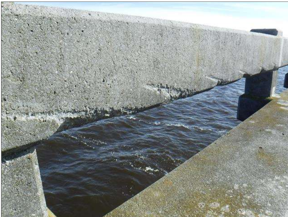
Span 168 Left Bridge Rail: 8' X 3" X 3" DAMAGED AREA AT BOTTOM RIGHT CORNER LOCATED ON RAILING BETWEEN 7 AND 8
