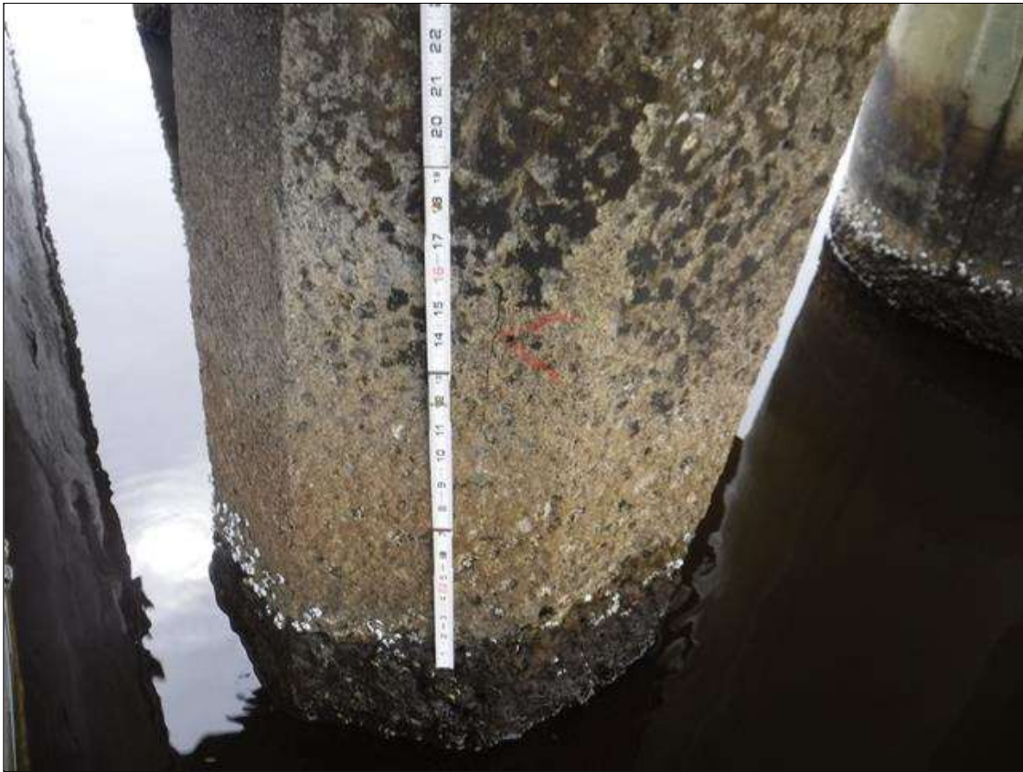
Bent 235 Pile 5: (PAR) (2) UP TO 3' X 0.03" VERTICAL CRACKS, BEGINNING 8' BOTTOM OF CAP, AT RANDOM THROUGHOUT.
