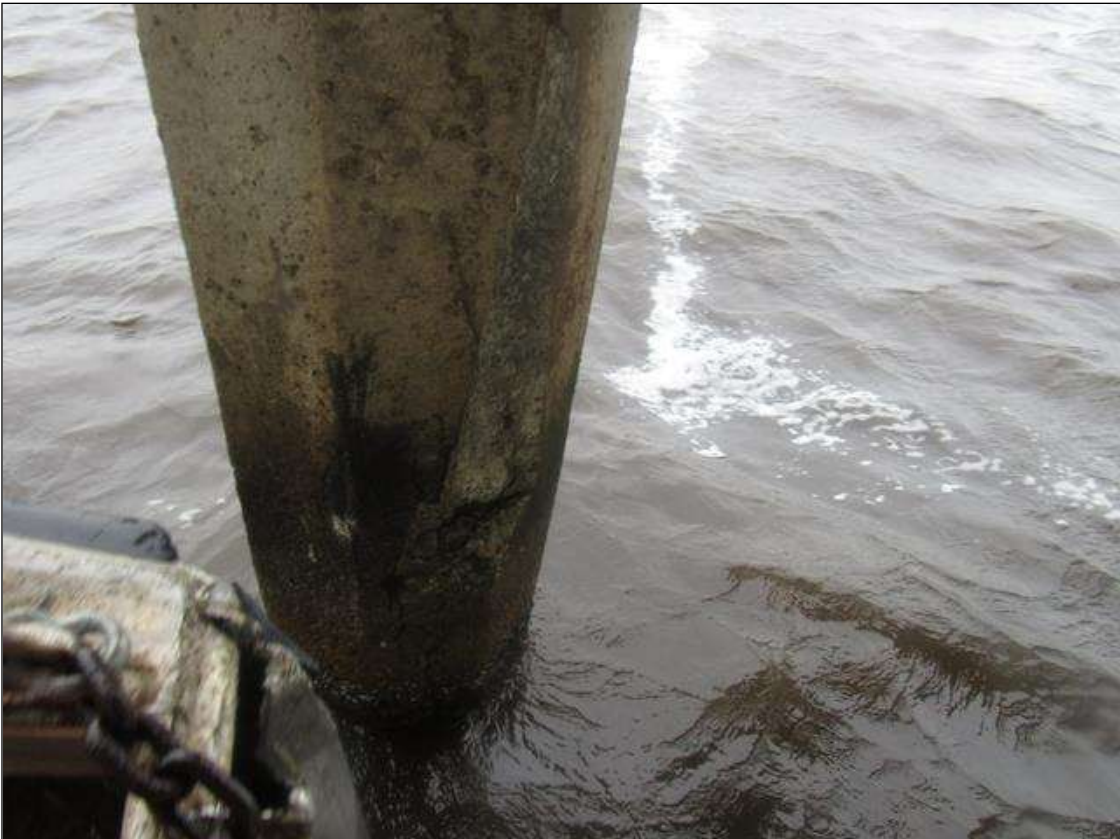
Bent 105 Pile 1: (PAR) 3' X UP TO 10" X 2" SPALL WITH EXPOSED REINFORCING AND SURROUNDING 3' OF DELAMINATION, SOUTH FACE, 9' FROM BOTTOM OF CAP.
