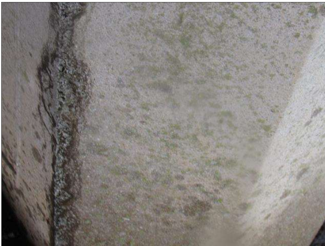
Bent 70 Pile 2: DELAMINATION 3' X 1' ON NORTH AND SOUTH FACES 8' FROM BOTTOM OF CAP
