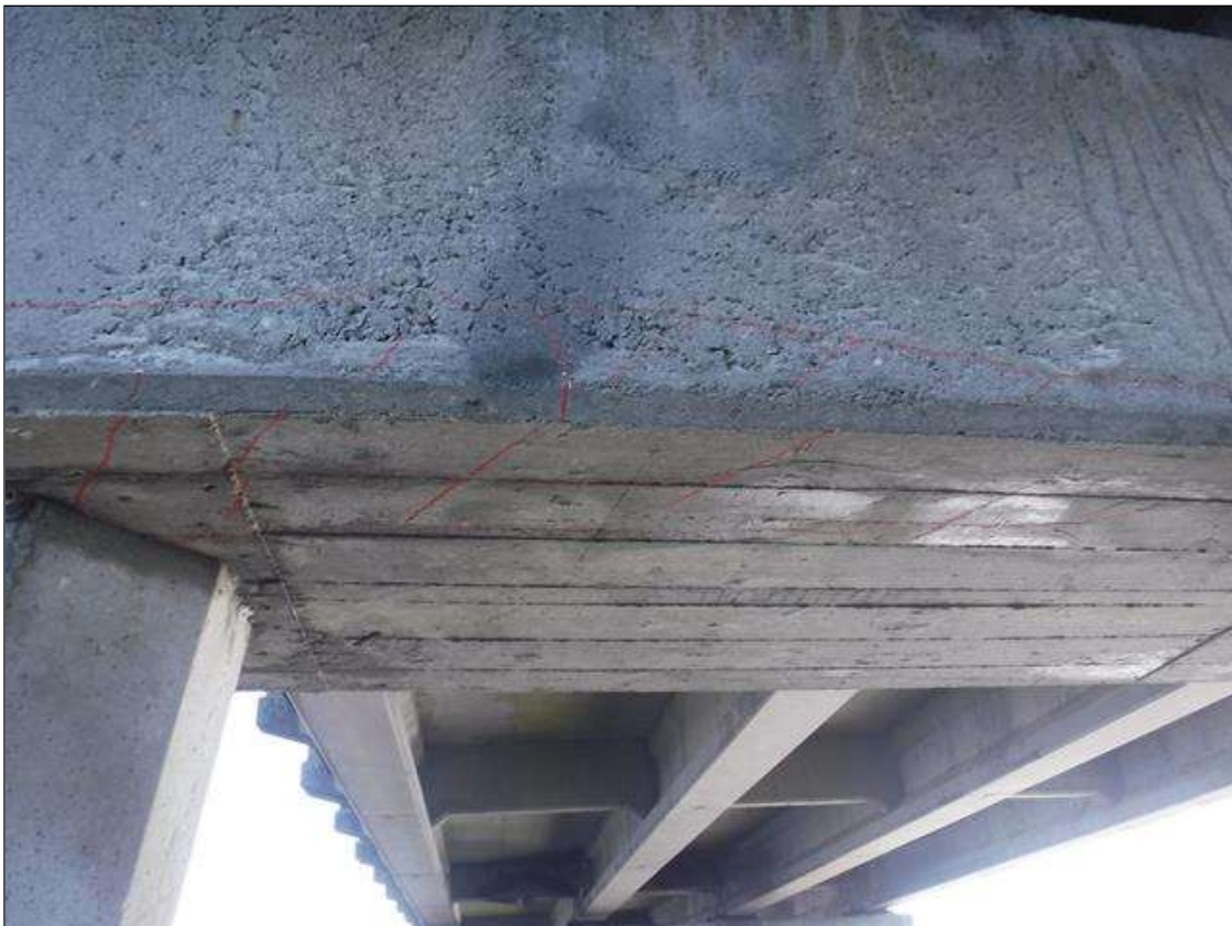
Bent 161 Cap 1: 6' LONG X 6" HIGH X 18" DEEP DELAMINATION AND SPALL ON BOTTOM WEST OF CAP, STARTING 1' FROM NORTH FACE.
