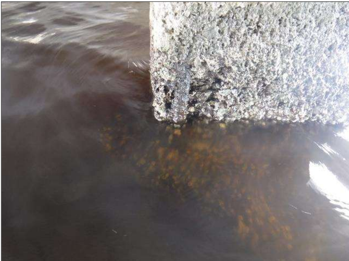
Bent 296 Pile 3: (PAR) 8" X 5" X 5" SPALL, WITH EXPOSED PRIMARY REINFORCING, NORTHWEST CORNER, 2' FROM BOTTOM OF CAP. REBAR HAS 5% SECTION LOSS
