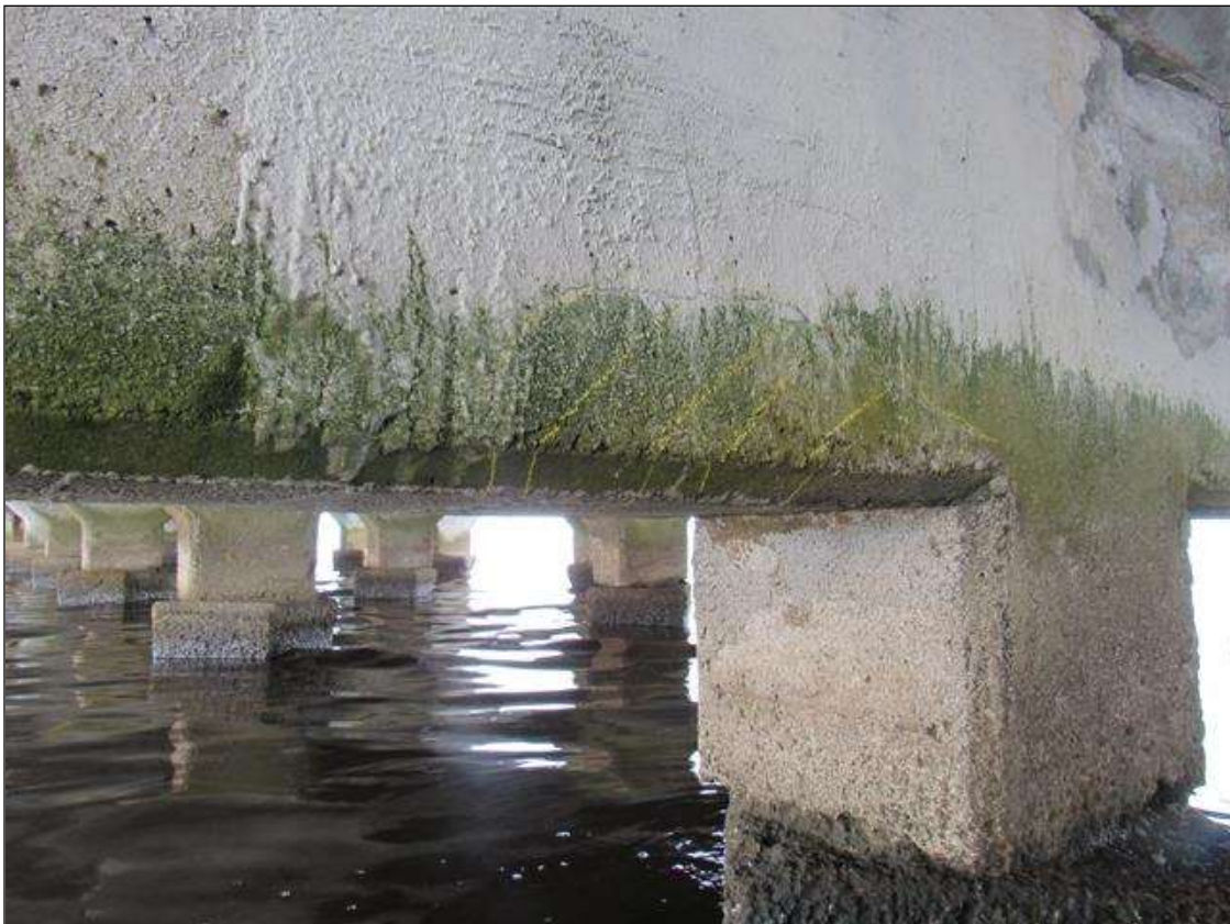
Bent 283 Cap 1: 8" X 22" DELAMINATION ON EAST FACE AT BOTTOM CORNER, BAY 3
