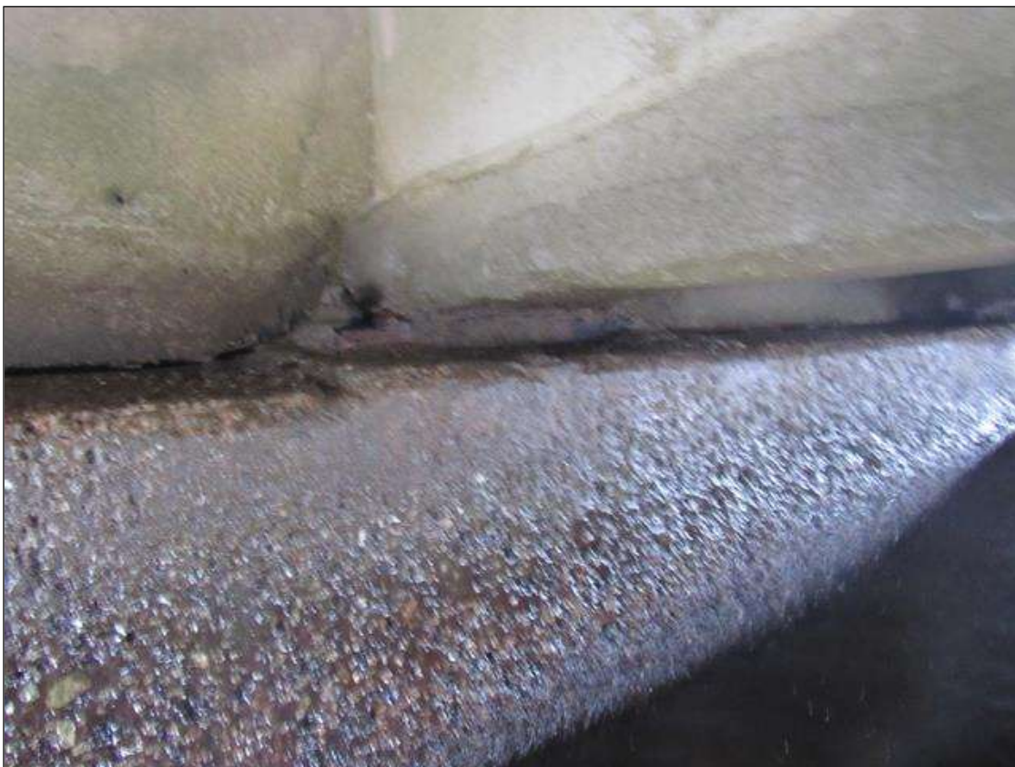
TYPICAL END BENT BEARING, END BENT 1 BEAM 3 SHOWN
