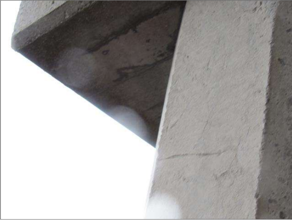
Bent 104 Pile 1: 5' X 9' AREA OF UP TO 0.009" MAP CRACKING, WEST FACE, BEGINNING AT BOTTOM OF CAP.
