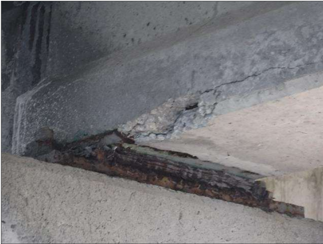
Span 19 Beam 3: 12" X 2" X 3" CORNER SPALL ADJACENT TO A 12" X 8" DELAMINATION, BOTTOM FACE, AT BENT 19.
