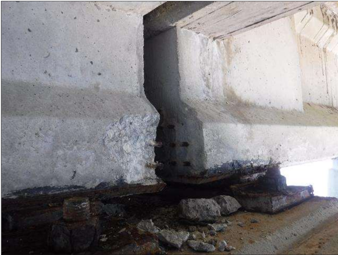
Span 132 Beam 3: (PAR) 6" X 6" X 2" DEEP SPALL WITH EXPOSED STRAND ON SOUTH FACE AT BENT 132
