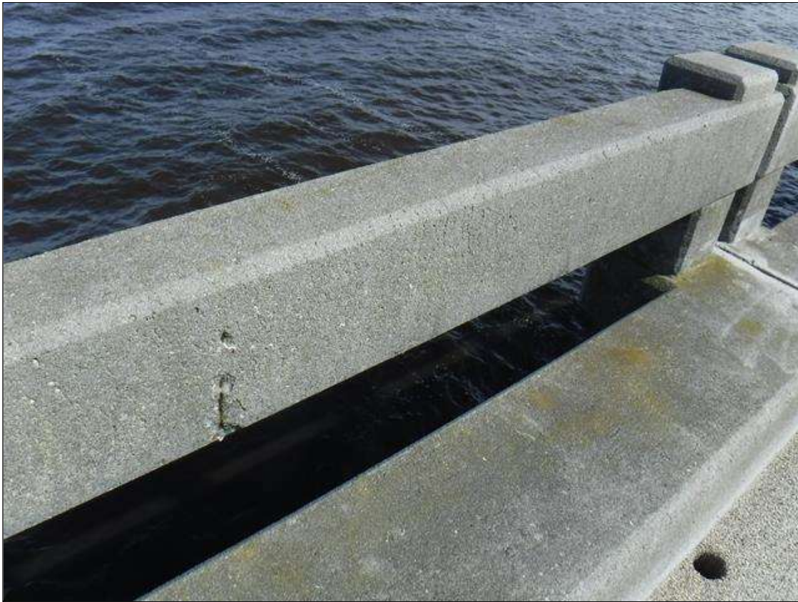
Span 191 Left Bridge Rail: 9" X 2" X 1/2" SPALL ON RIGHT FACE LOCATED ON RAILING 30" FROM POST 8
