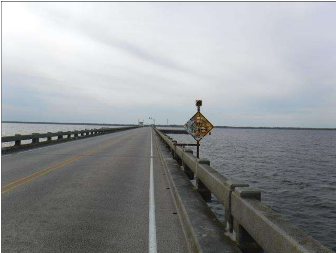
(PAR) DRAW BRIDGE SIGNS ON RIGHT SIDE OF SPAN 99 AND LEFT SIDE OF SPAN 133 ARE OBSTRUCTED FROM VIEW
