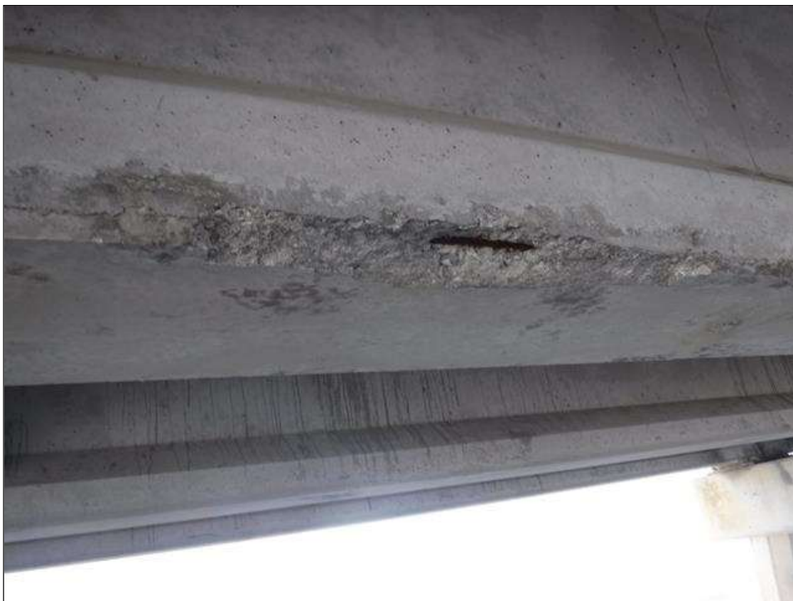
Span 73 Beam 2: (PAR) 3' X 2" HIGH X 4" DEEP SPALL WITH EXPOSED STRAND ON BOTTOM AND NORTH FACE AT MIDSPAN
