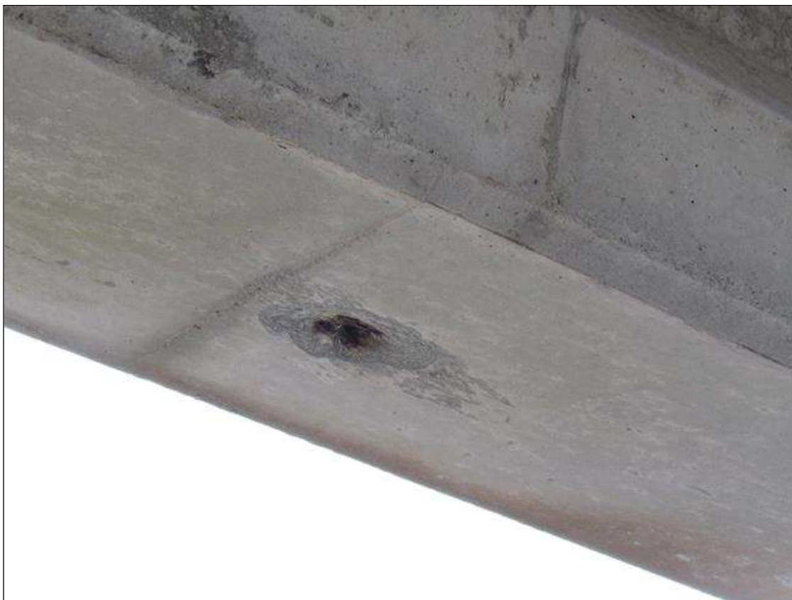
Span 33 Beam 1: 3" DIAMETER X 1/2" DEEP SPALL ON BOTTOM FACE AT MIDSPAN
