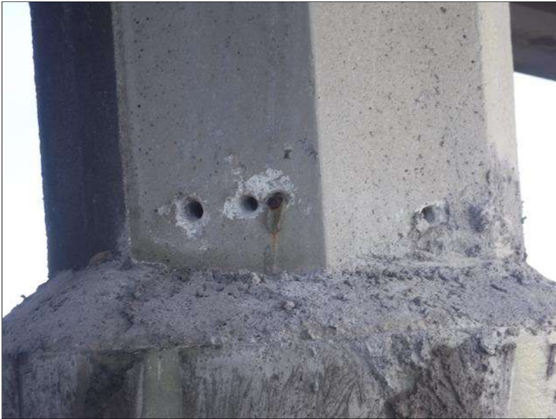
Bent 155 Saved Pile 5: (3) 1/2" DIAMETER HOLES, WITH EXPOSED STRANDS, SOUTH FACE, 2' FROM BOTTOM OF CAP.
