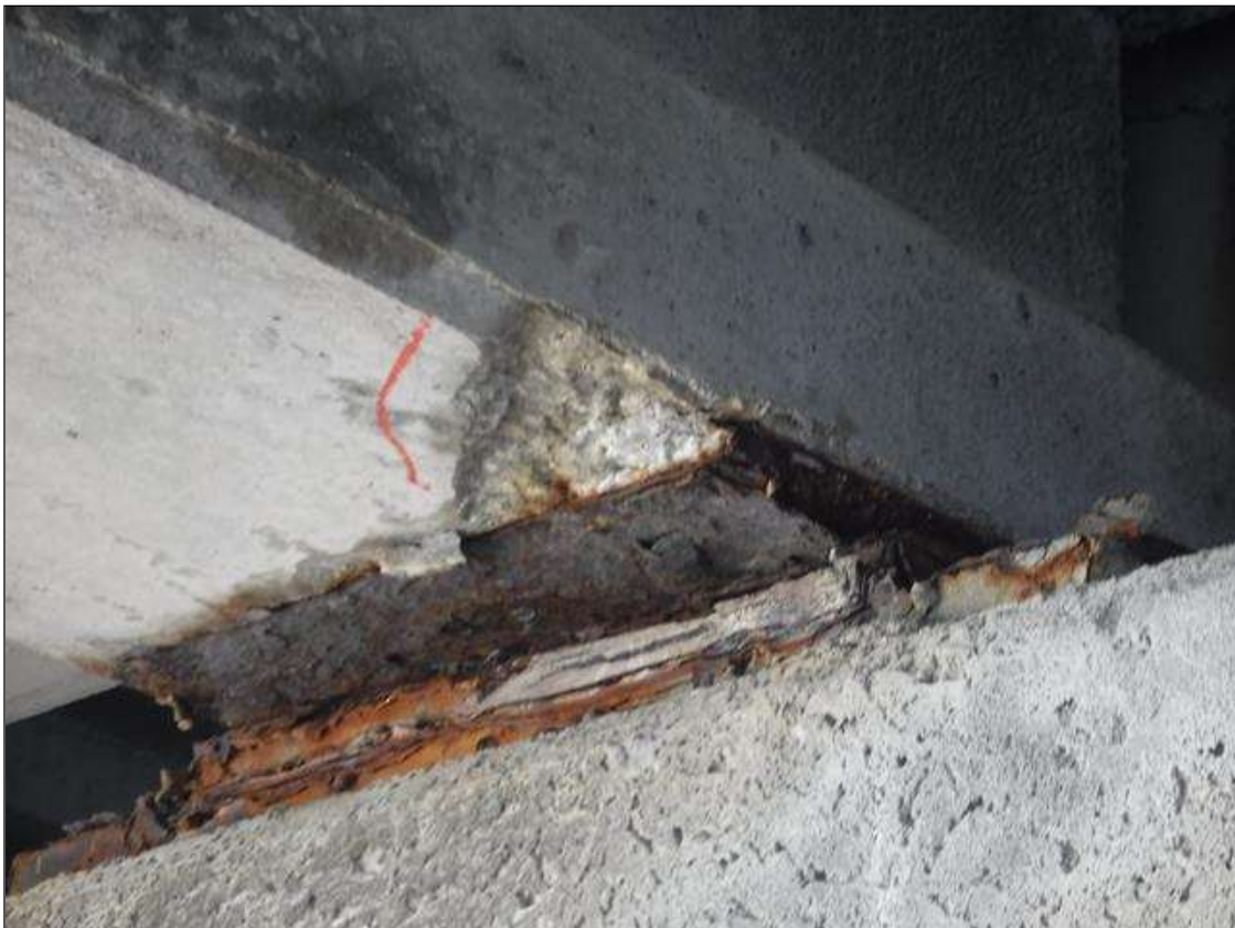
Span 161 Beam 3: 6" DIAMETER X 3/4" DEEP SPALL IN BOTTOM FACE AT BENT 160
