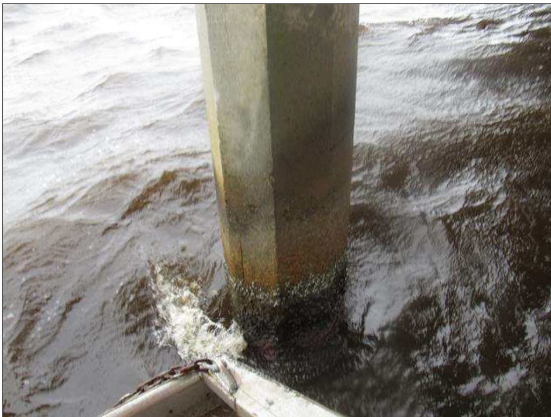
Bent 75 Pile 1: (PAR) UP TO 18" X 0.06" VERTICAL CRACKS, WEST FACE, BEGINNING 10' FROM BOTTOM OF CAP.
