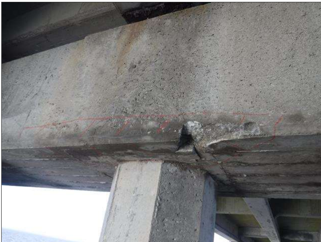
Bent 153 Cap 1: 4' LONG X 6" HIGH X 1' DEEP DELAMINATION WITH SPALL ON EAST FACE ABOVE PILE 3
