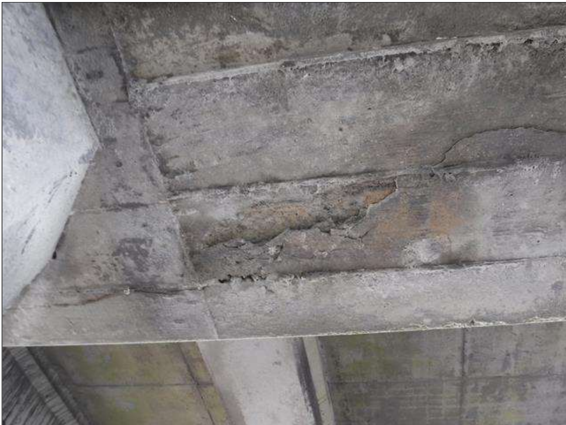
Bent 173 Cap 1: 8" X 2" X 1/2" SPALL, BOTTOM FACE, BETWEEN PILES 1 AND 2, NEAR PILE 2.
