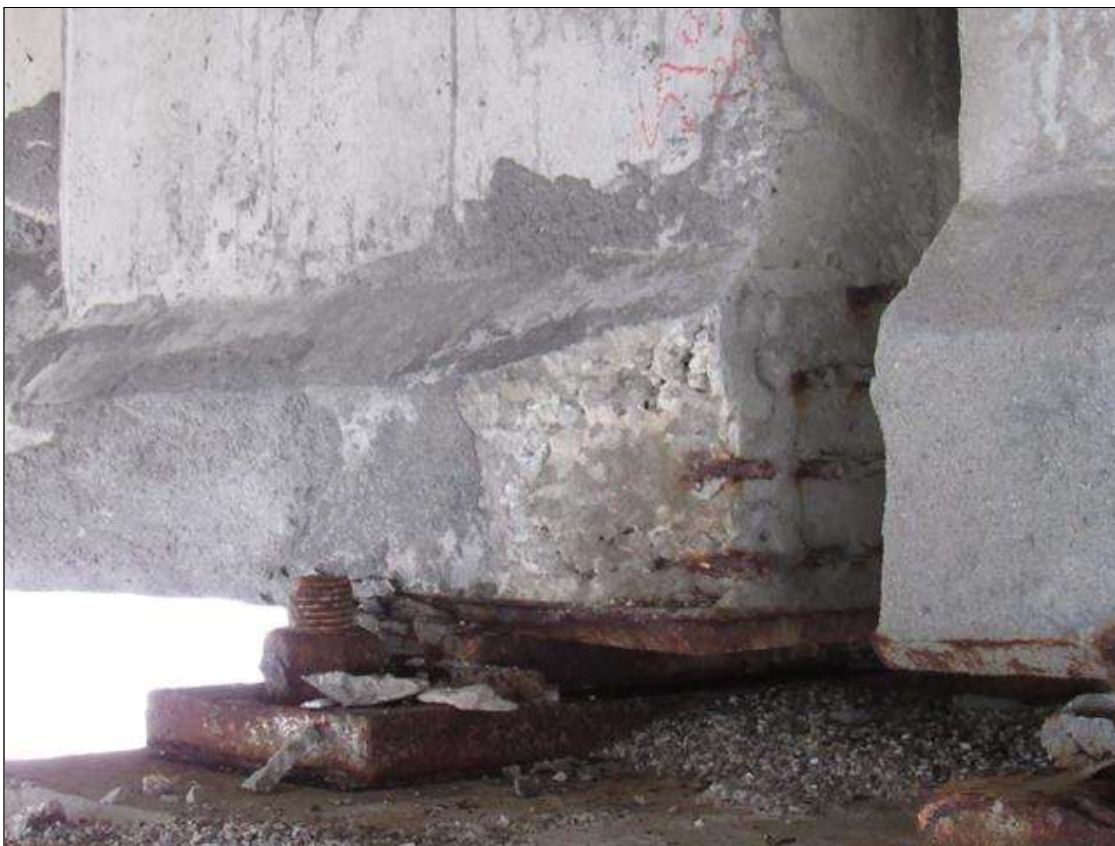
Span 70 Beam 2: 12" X 12" FAILED PATCH ON NORTH FACE AT BENT 69
