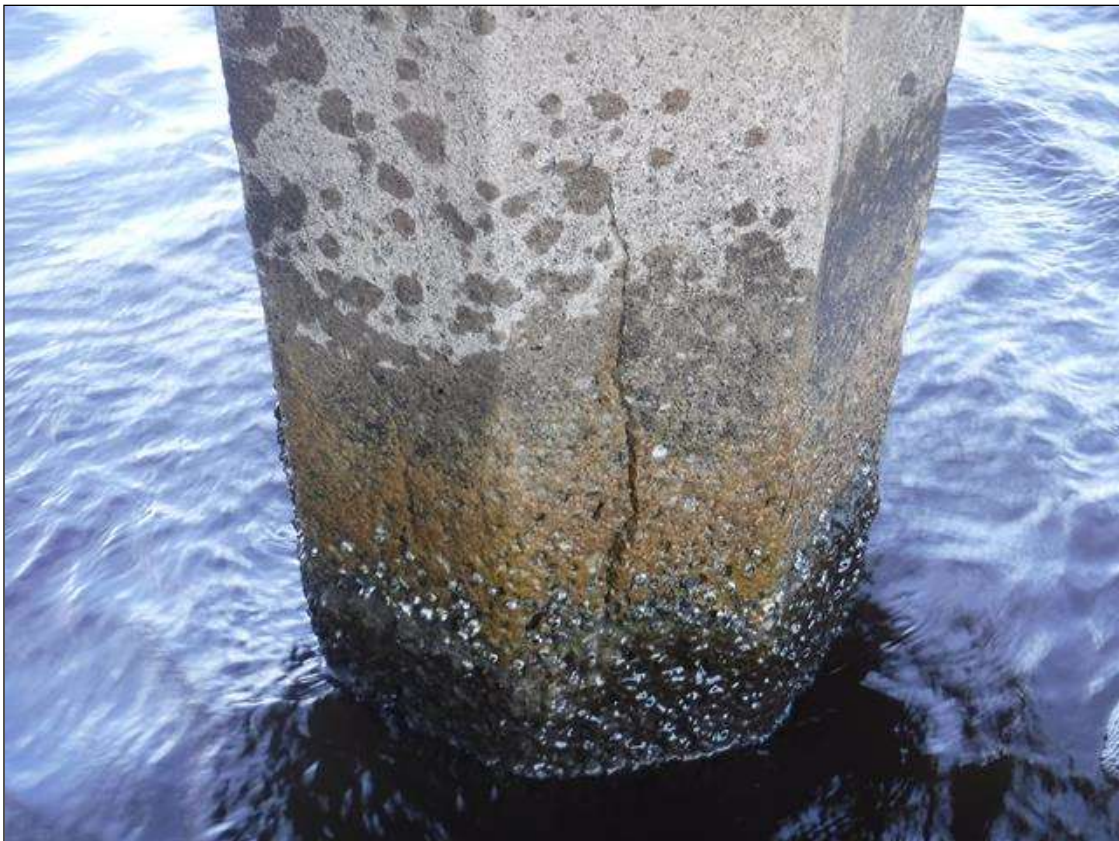
Bent 28 Saved Pile 1: (PAR) H/L TO 1/8" CRACK, 8' BELOW CAP, DOWN 6', SOUTH QUAD. SCALING TO 1" DEEP FROM WATERLINE TO MUDLINE.
