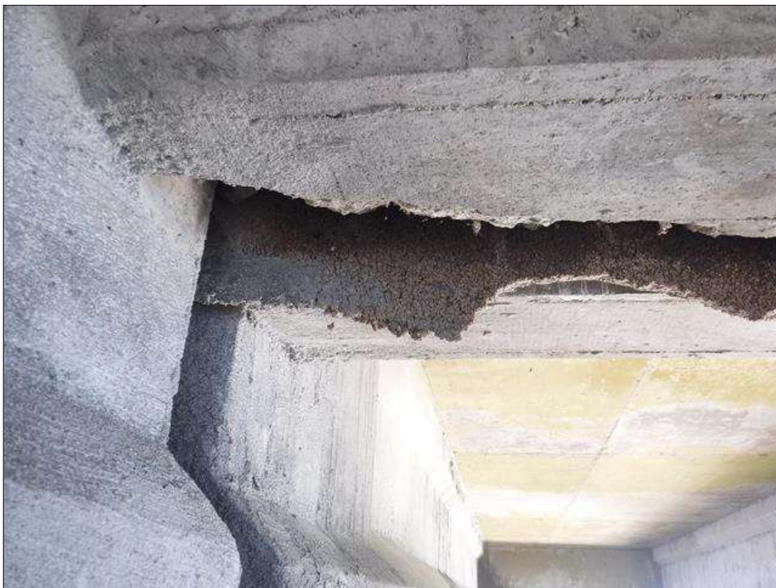
Span 137 Beam 3: 1.5' X 6" X 4" DEEP SPALL WITH EXPOSED REBAR ON EAST FACE BAY 3 DIAPHRAGM
