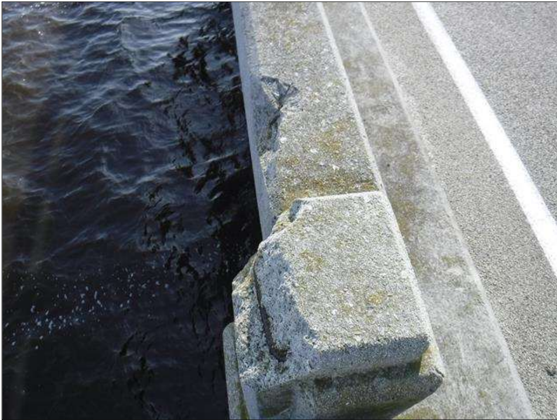
Span 137 Left Bridge Rail: 2' X 4" X 11" SPALL WITH EXPOSED REBAR AT TOP LEFT CORNER LOCATED ON POST 7 AND RAIL
