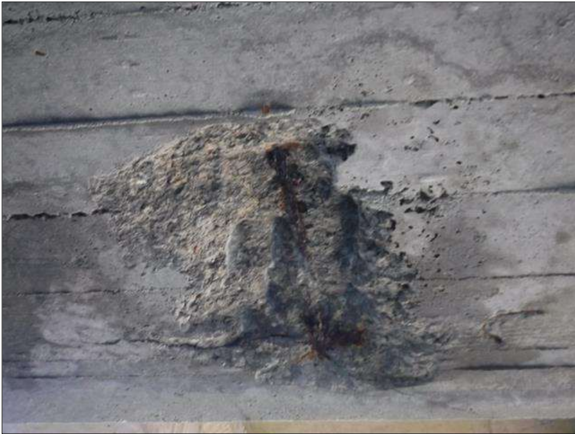
Bent 15 Cap 1: (PAR) 18" X 18" X UP TO 5" SPALL, WITH EXPOSED REINFORCING WITH COMPLETE SECTION LOSS, BOTTOM FACE, BETWEEN BEAMS 1 AND 2.
