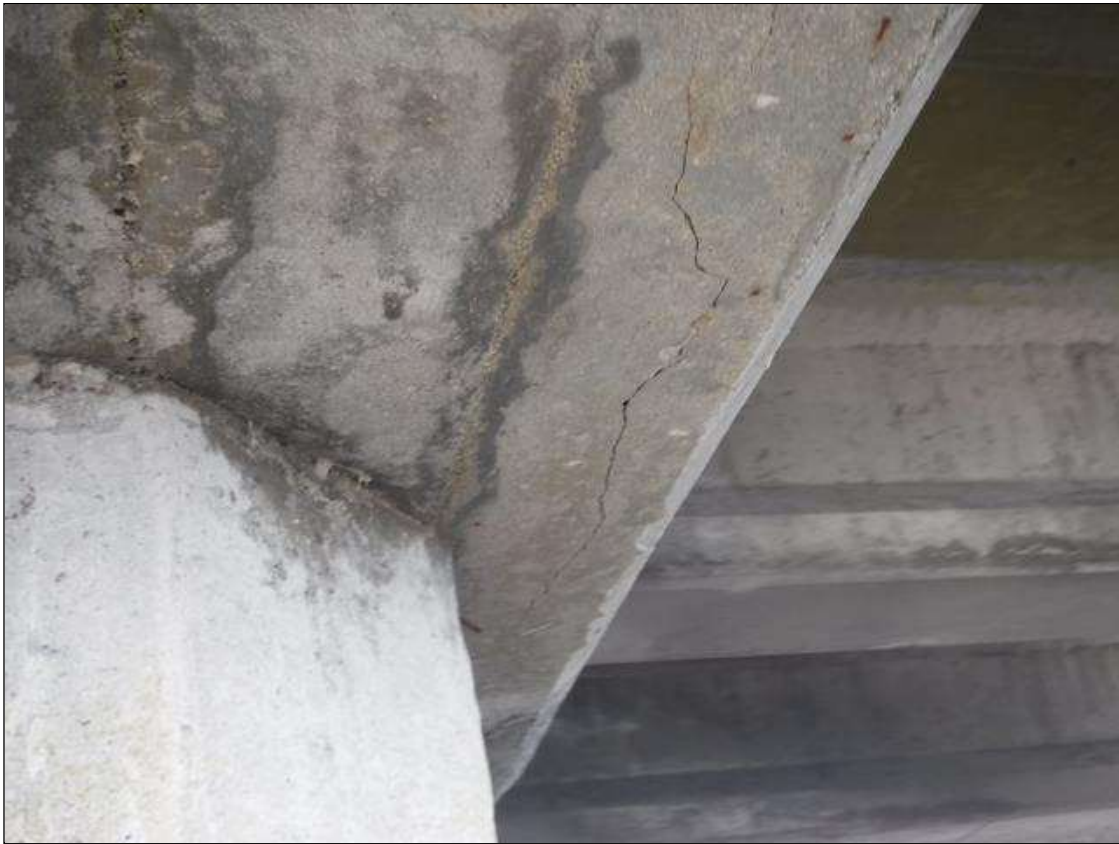
Bent 181 Cap 1: 3' LONG X 1/16" CRACK IN BOTTOM FACE EAST OF PILE 4
