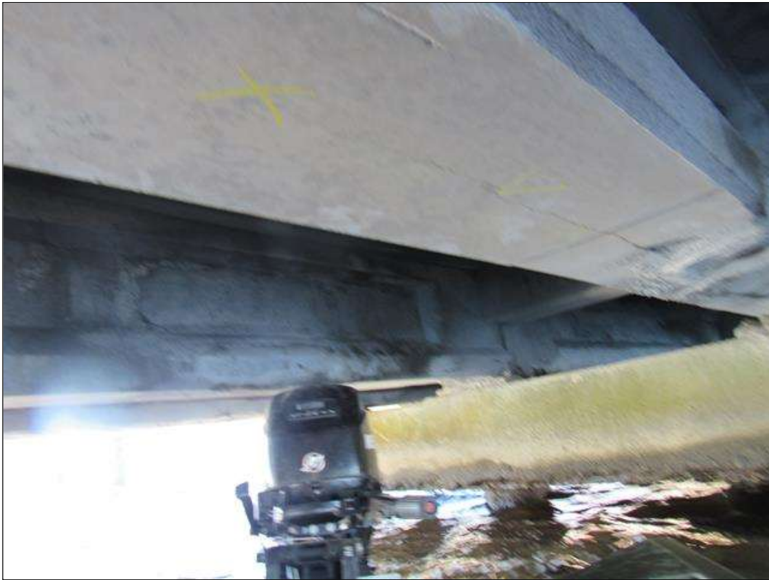
Span 3 Beam 2: (PAR) 3' X UP TO 0.031" LONGITUDINAL CRACK, BOTTOM FACE, 15' FROM BENT 2.
