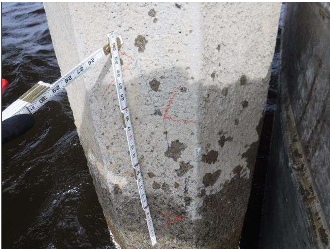
Bent 173 Pile 4: (PAR) (2) UP TO 6' X 0.063" VERTICAL CRACKS, SOUTH FACE, BEGINNING 8' FROM BOTTOM OF CAP.
