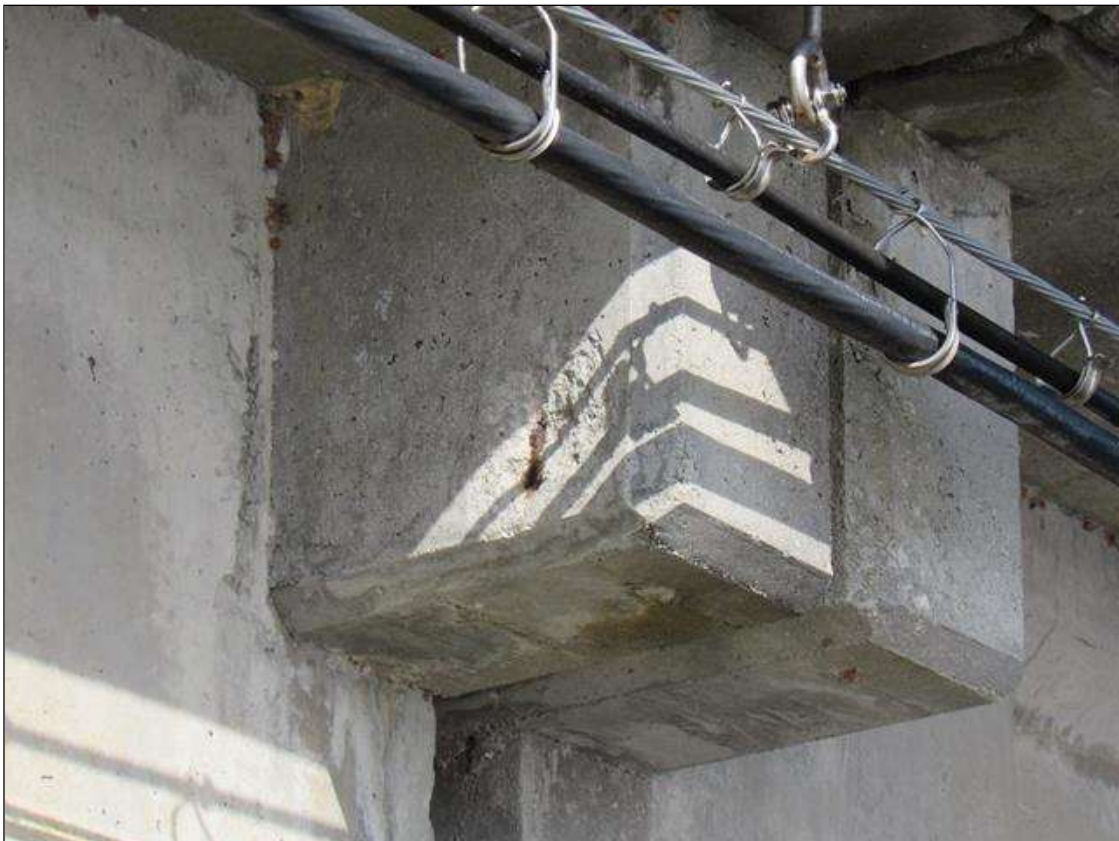
Span 6 Beam 4: 6" X 6" X 1" SPALL, WITH EXPOSED REINFORCING, WEST FACE OF BENT 6 SOUTH OVERHANG DIAPHRAGM.
