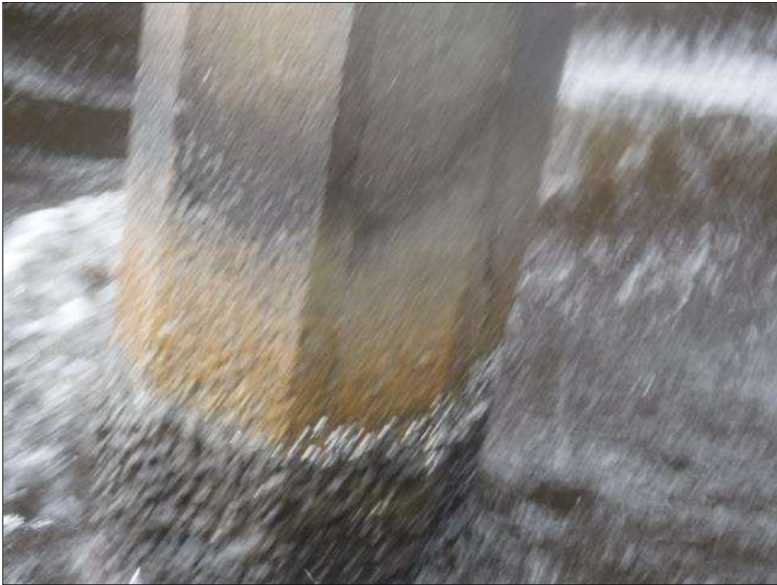
Bent 88 Pile 1: (PAR) UP TO 3' X 0.06" VERTICAL CRACKS WITH 4' X 2' DELAMINATION ON NORTH AND WEST FACE, BEGINNING 8' BOTTOM OF CAP.
