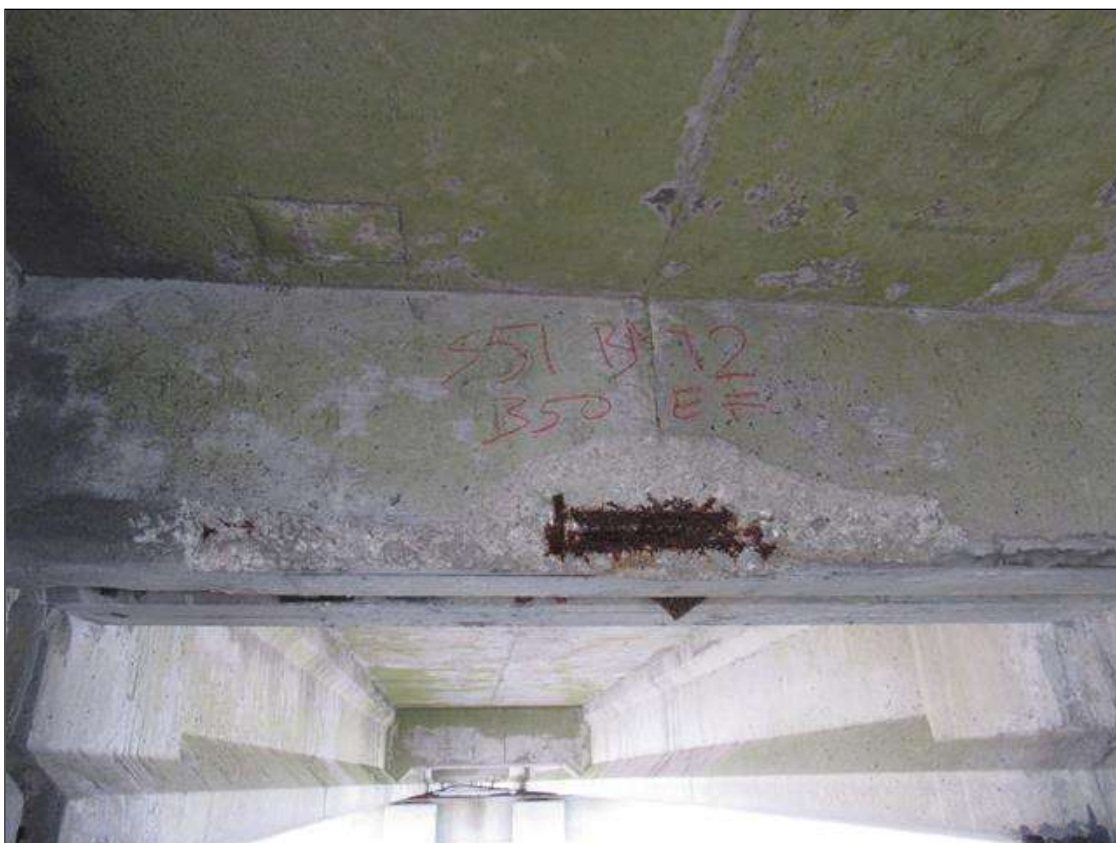
Span 51 Beam 2: 45" X 7" HIGH x 4" DEEP SPALL WITH 12" OF EXPOSED REBAR ON END DIAPHRAGM IN BAY 2 AT BENT 50
