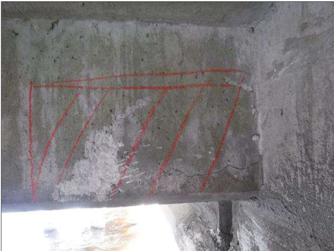
Span 147 Beam 3: 2' X 2' DELAMINATION, WEST FACE OF BENT 147 DIAPHRAGM, BETWEEN BEAMS 2 AND 3
