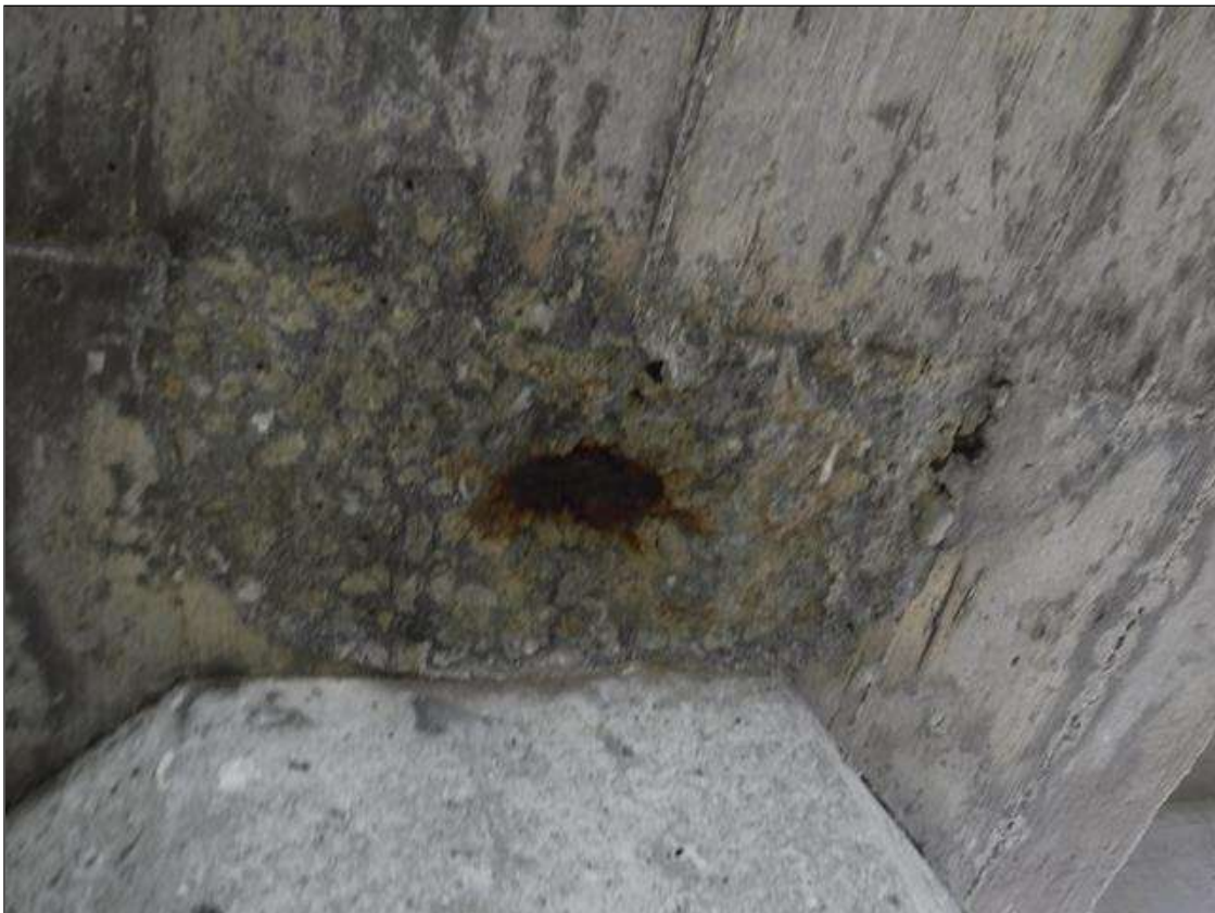
Bent 188 Cap 1: 6" X 12" X 1/2" SPALL, WITH EXPOSED REINFORCING, BOTTOM FACE, BETWEEN BEAMS 2 AND 3, AT BENT 188.
