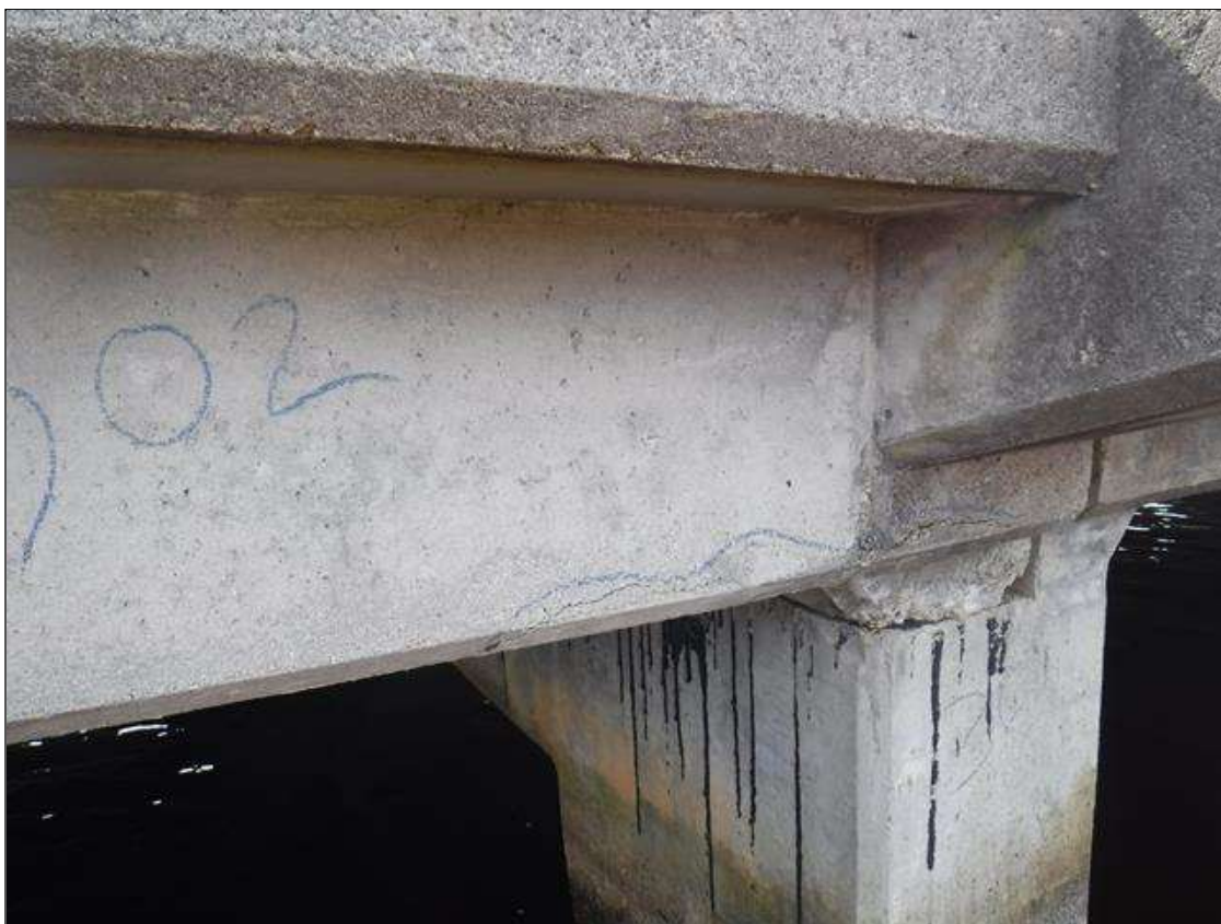
Span 302 Left Bridge Rail: 2' X UP TO 1/16" WIDE LONGTINUAL CRACK AT BOTTOM LEFT CORNER AT BENT 301
