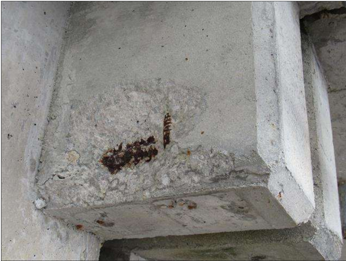
Span 55 Beam 4: 12" X 8" X 1" DEEP SPALL WITH EXPOSED REBARS ON END DIAPHRAGM AT SOUTH OVERHANG AT BENT 55
