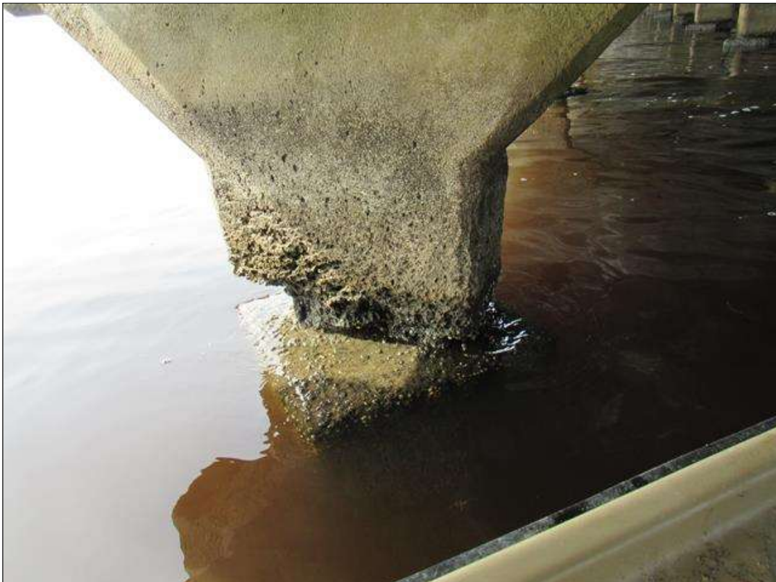
Bent 288 Pile 4: (PAR) 12" X 20" X 10" SPALL, WITH EXPOSED REBAR, EAST FACE, 2' FROM BOTTOM OF CAP.
