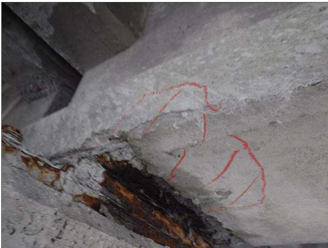
Span 179 Beam 2: 10" X 10" X 4" DELAMINATION ON BOTTOM FLANGE SOUTH FACE AT BENT 178
