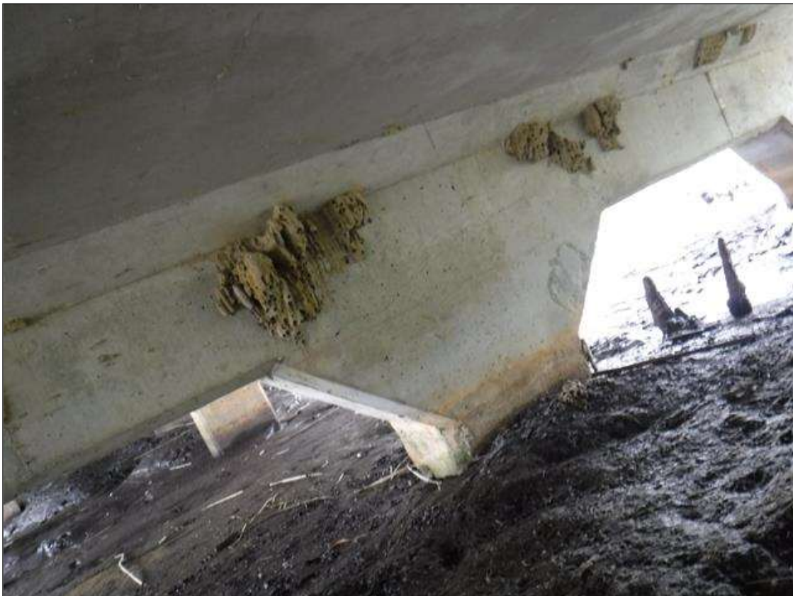
Bent 342 Cap 1: 4' LONG X UP TO 1/16" WIDE LONGITUDINAL CRACK ON EAST FACE LOCATED ABOVE PILE 2
