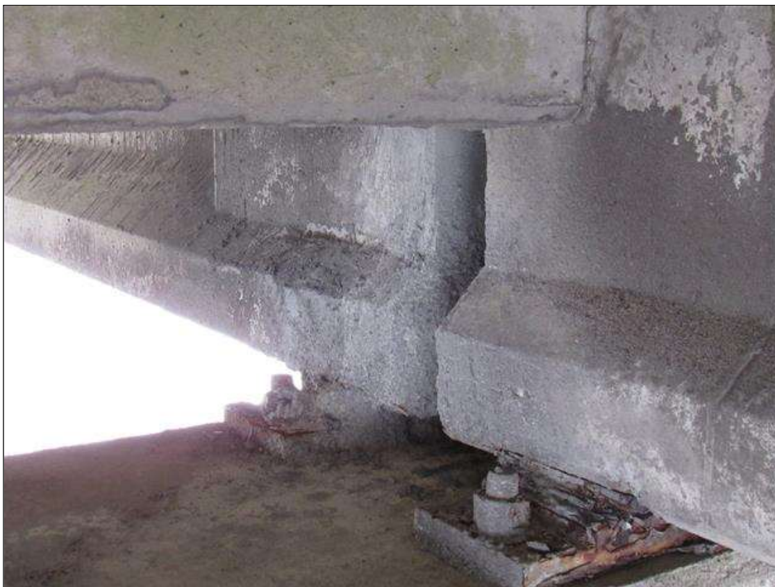
Span 44 Beam 3: 3' X UP TO 5" PATCHED AREA, BOTTOM FACE, EXTENDING 1' ONTO NORTH FACE, AT BENT 43.
