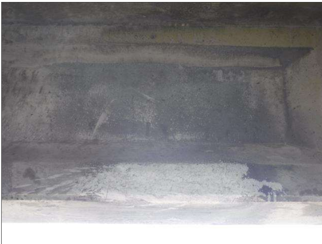
Span 154 Beam 4: 3' X UP TO 1' X 4" CRACKED PATCHED AREA UP TO 0.031", NORTH FACE, 3' FROM BENT 153
