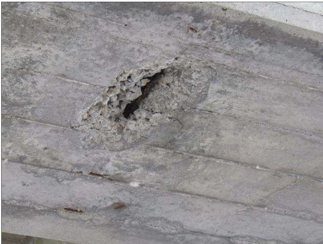
Bent 40 Cap 1: 9" X UP TO 12" X 1" SPALL, WITH EXPOSED REINFORCING, BOTTOM OF CAP, BETWEEN PILES 2 AND 3.
