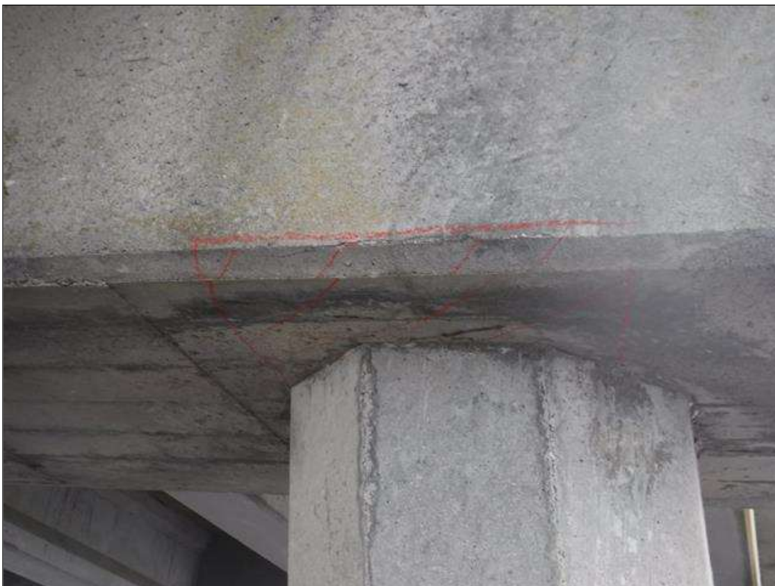
Bent 242 Cap 1: 2' X 18" DELAMINATION ON BOTTOM FACE AT PILE 6
