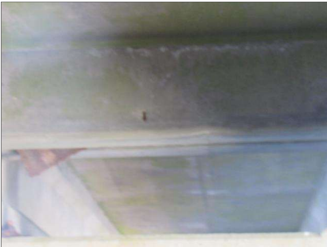
Span 6 Beam 1: 2" X 2" X 1/2" SPALL, WEST FACE OF BENT 6 DIAPHRAGM, BETWEEN BEAMS 1 AND 2.
