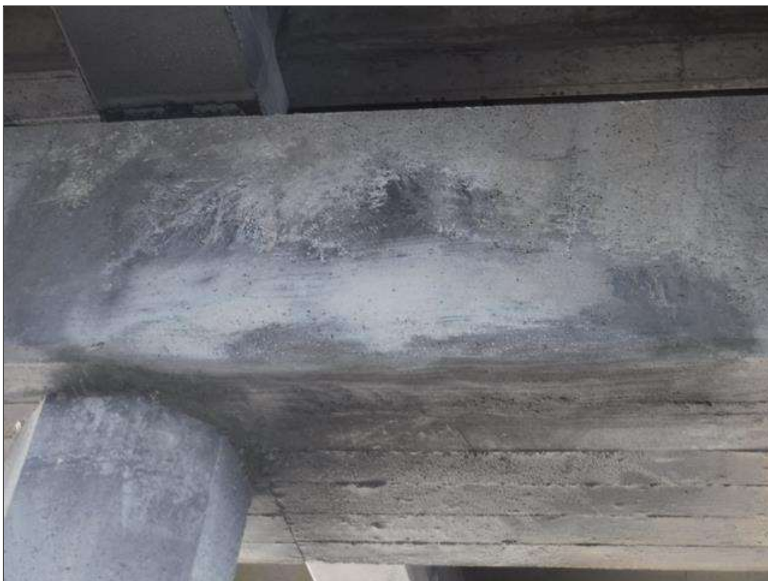
Bent 126 Cap 1: 3' X 18" PATCHED AREA, EAST FACE, ABOVE PILE 3
