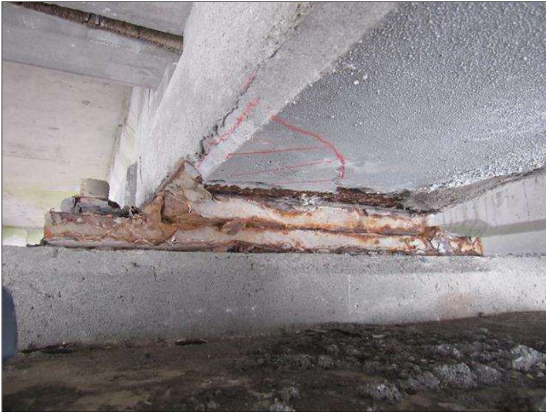
Span 34 Beam 3: 4' X UP TO 8" PATCHED AREA WITH 7" X 8" DELAMINATION, BOTTOM FACE, EXTENDING 1' ONTO NORTH FACE, AT BENT 33.
