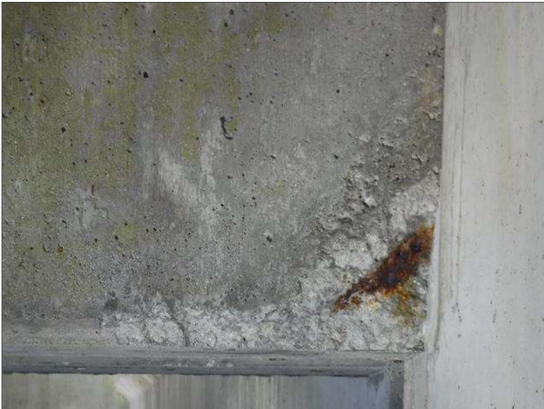
Span 137 Beam 3: 1' DIAMETER X 1" DEEP SPALL WITH EXPOSED REBAR ON EAST FACE BAY 3 DIAPHRAGM
