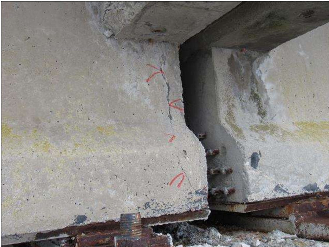
Span 55 Beam 4: (PAR) 16" LONG X UP TO 1/16" WIDE VERTICAL CRACK ON SOUTH FACE AT BENT 55
