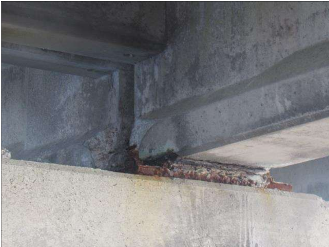
Span 8 Beam 3: (PAR) 6" X 10" X 3" SPALL WITH EXPOSED STRAND, NORTH FACE, AT BENT 7.
