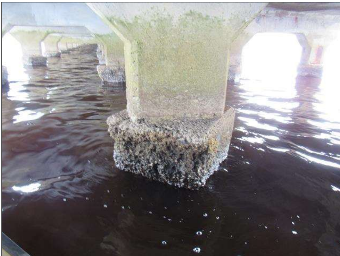
Bent 279 Pile 2: (PAR) 24" X UP TO 12" X UP TO 6" DEEP SPALL WITH EXPOSED REINFORCING ON WEST FACE ON PILE 2 FOOTING
