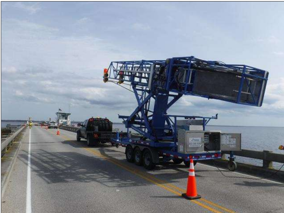
SNOOPER USED FOR SPANS 30-150 SUPERSTRUCTURE UNDERSIDE
