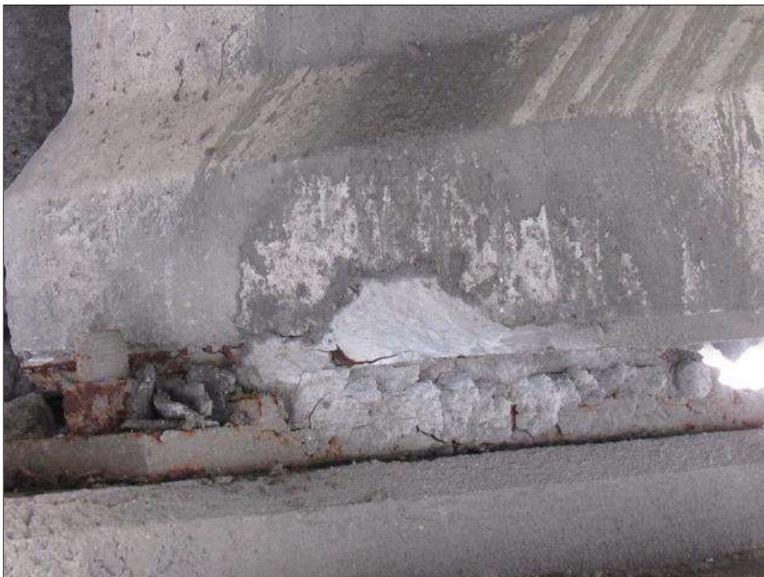
Span 49 Beam 3: 1' X UP TO 6" X 3" SPALL, BOTTOM FACE, AT BENT 49.
