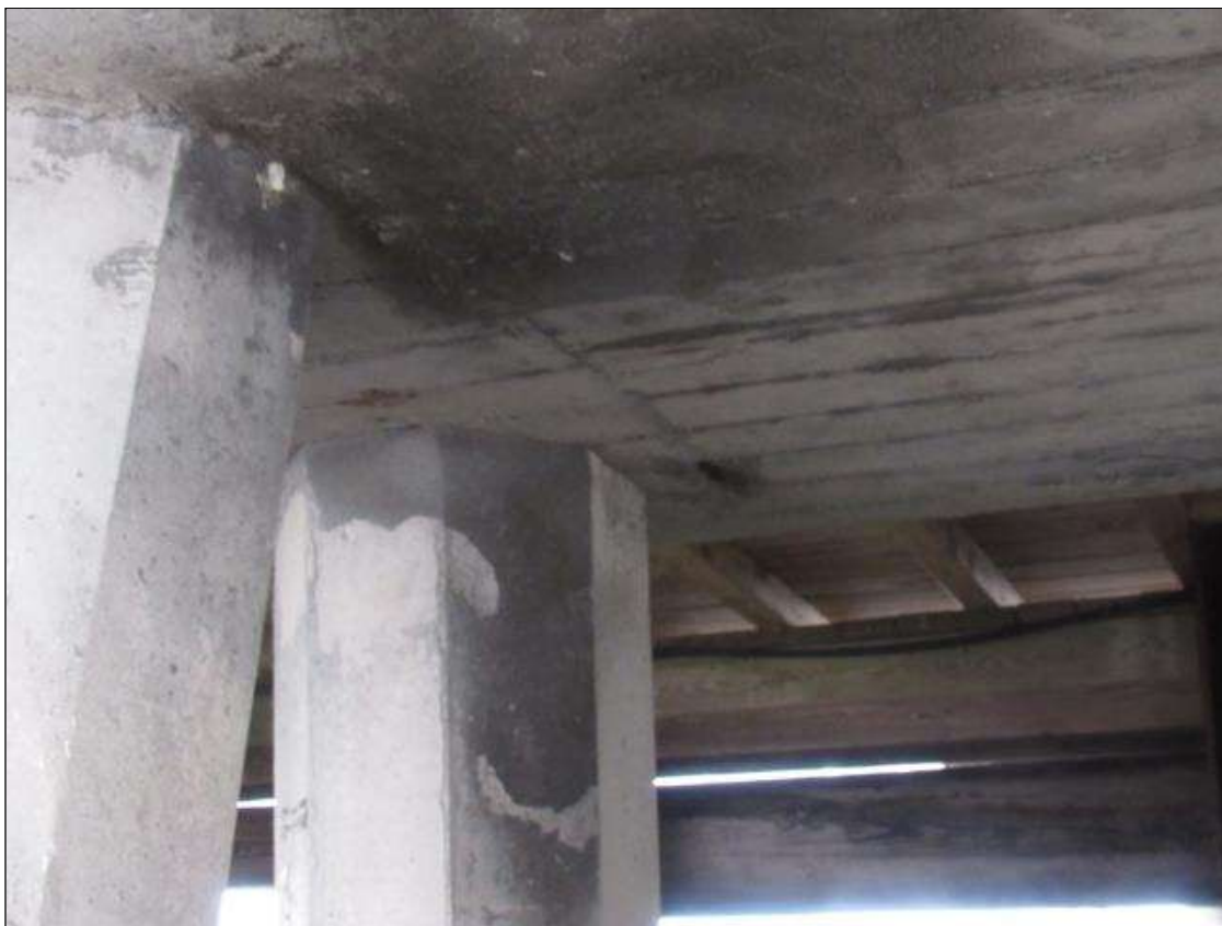
Bent 115 CAP REST PIER 1: 1' X 1' X 1" DEEP SPALL WITH EXPOSED REBAR AND 2' AREA OF SURROUNDING DELAMINATION BOTTOM FACE NEAR PILE 10
