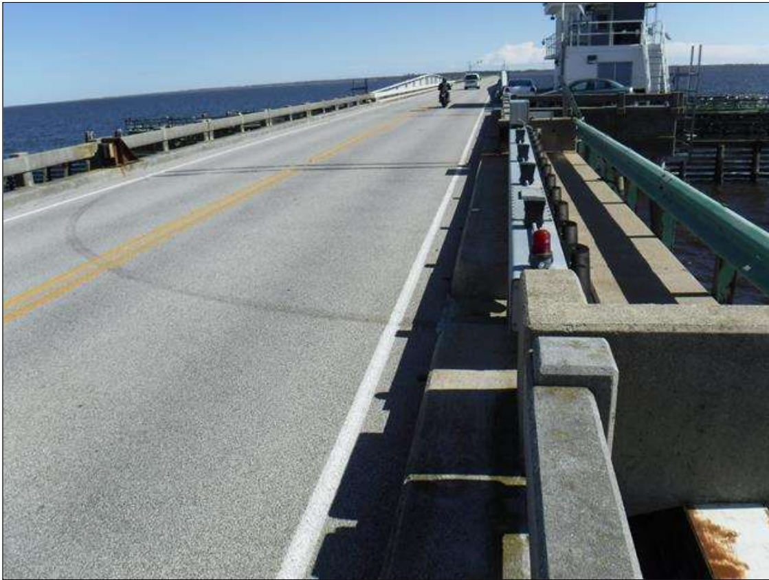
RIGHT SIDE CLOSURE GATE AT SPAN 113
