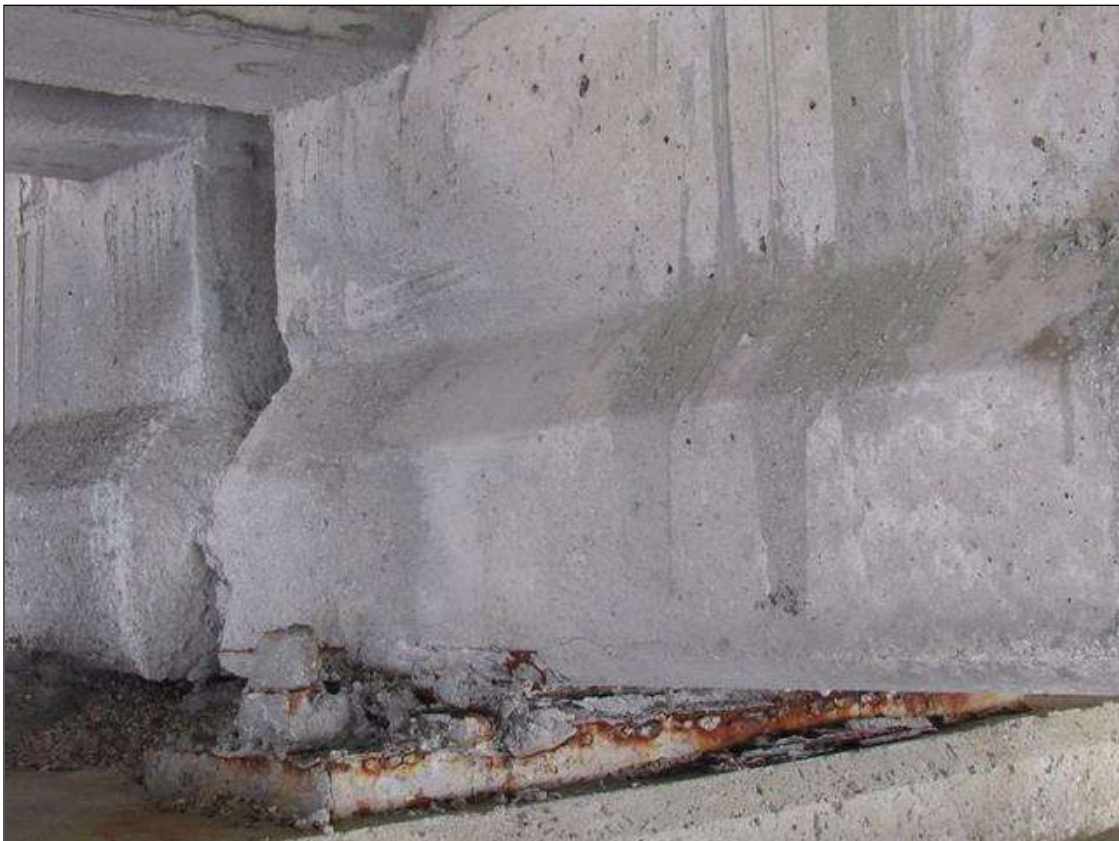
Span 61 Beam 3: (2) UP TO 12" X 12" PATCHED AREAS, NORTH AND SOUTH FACES, AT BENT 61.
