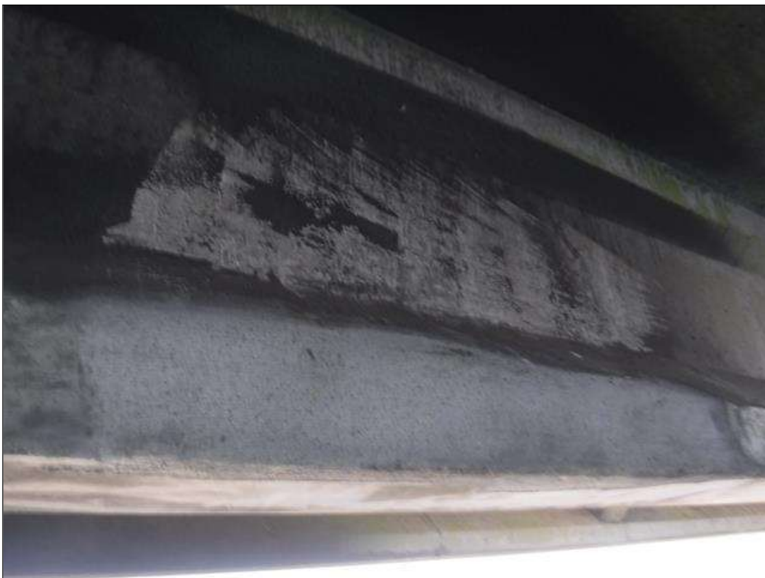
Span 9 Beam 3: 5' OF PATCHED AREA IN BOTTOM BULB OF GIRDER, 20' FROM BENT 9.
