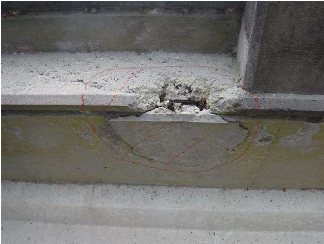
Span 234 Deck: (PAR) 3' X 6" X 2' DEEP SPALL WITH EXPOSED REBAR WITH UP TO 50% SECTION LOSS, ON DECK UNDERSIDE AT LEFT OVERHANG AT MIDSPAN
