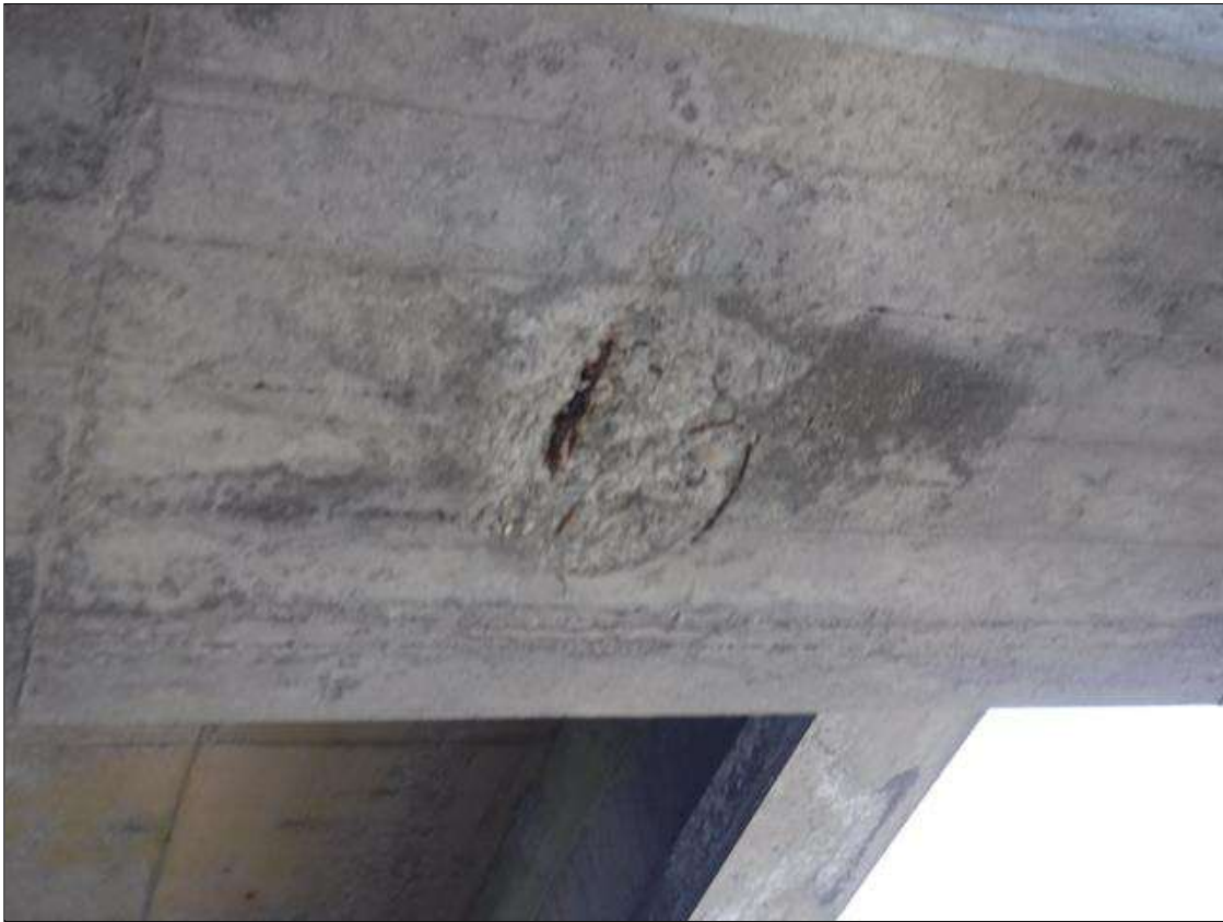
Bent 26 Cap 1: 12" X 12" X 2" SPALL, WITH EXPOSED REINFORCING, BOTTOM FACE, BETWEEN BEAMS 3 AND 4.
