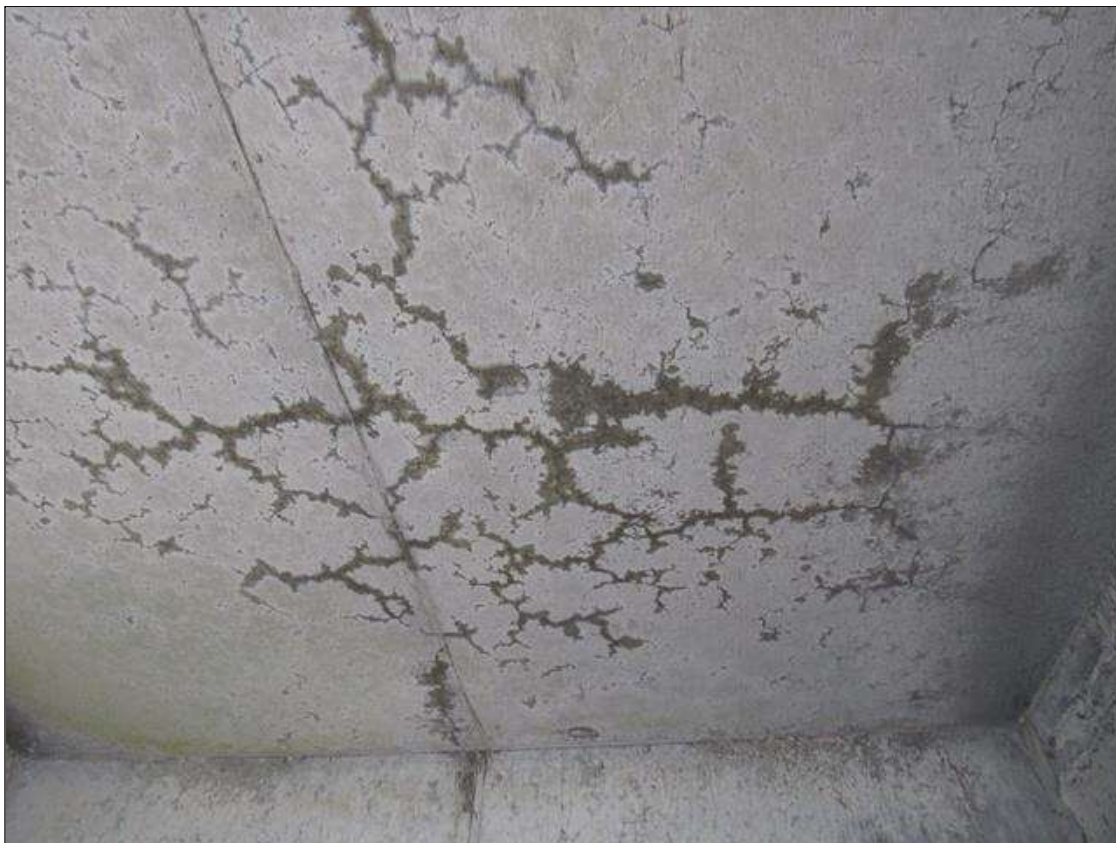
Span 65 Deck: 150 SF OF HAIRLINE MAP CRACKING, UNDERSIDE OF DECK
