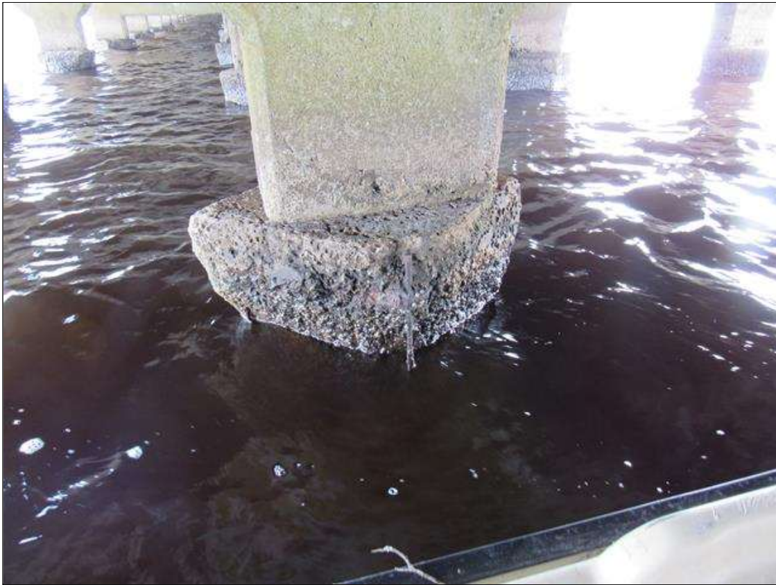
Bent 280 Pile 2: (PAR) 24" X 24" X 5" SPALL, WITH EXPOSED REBAR WITH COMPLETE SECTION LOSS TO VERTICAL BARS, WEST FACE OF COLUMN FOOTING.
