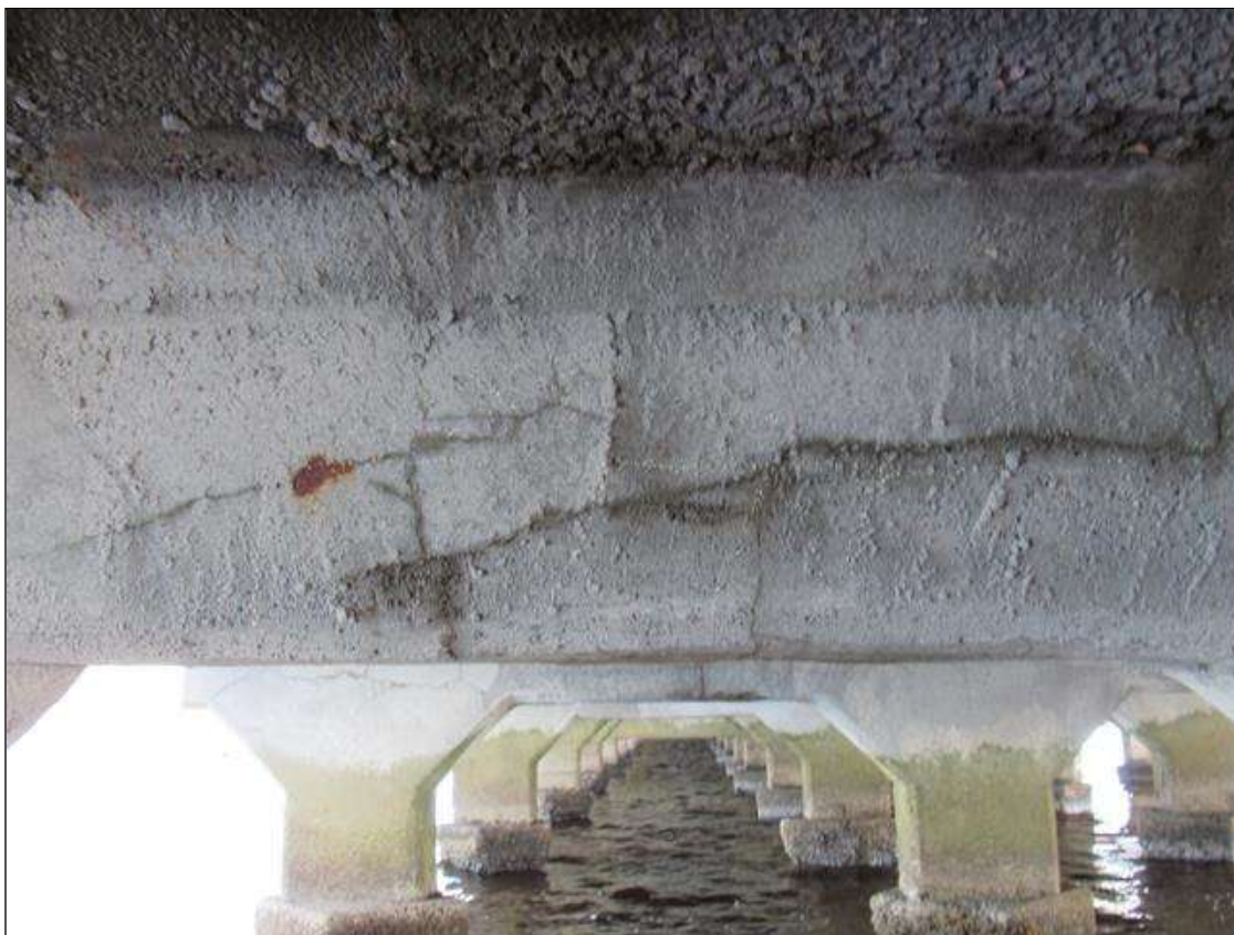
Bent 278 Cap 1: 3' X 1' CRACKED PATCHED AREA, WITH RUST STAINING, WEST FACE, BAY 1.
