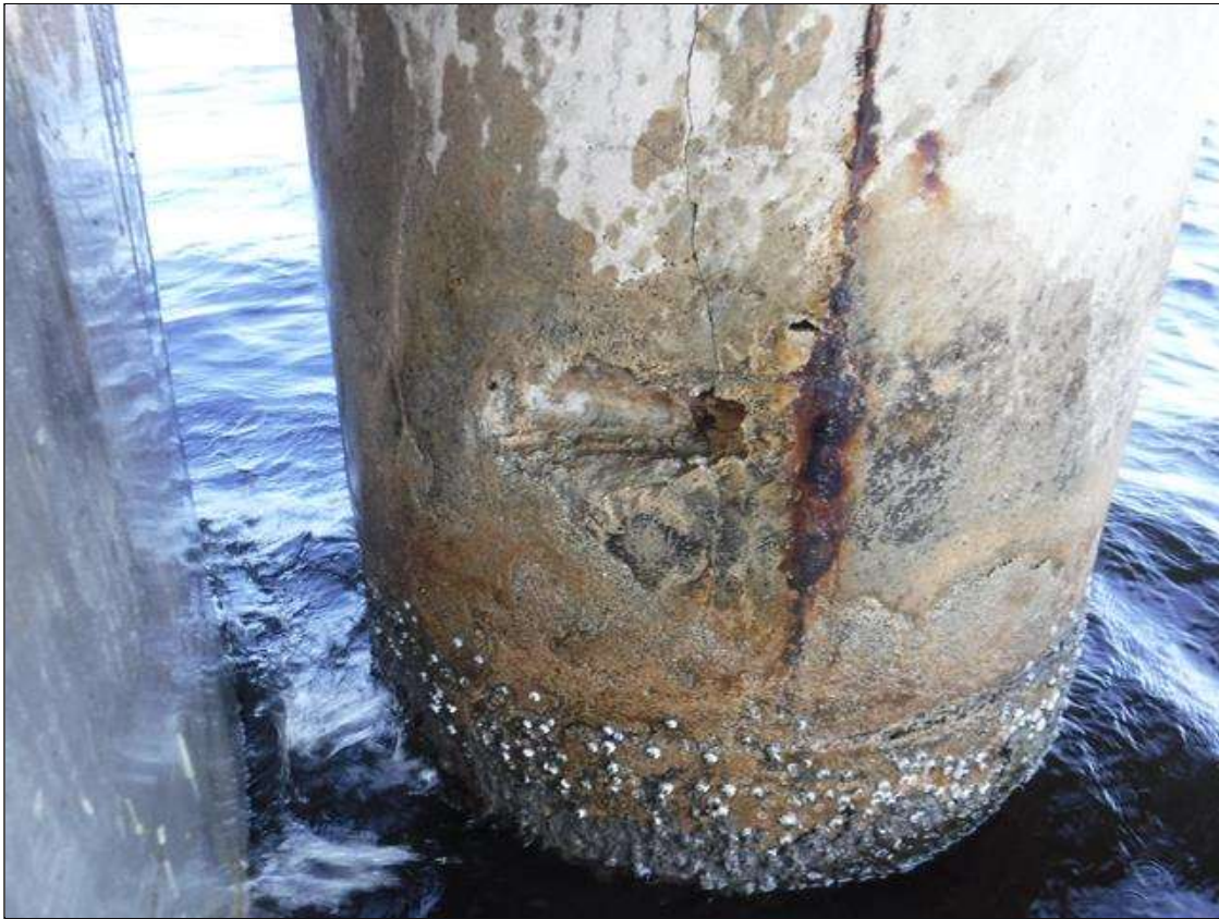
Bent 14 Saved Pile 2: 8" X 3" X UP TO 1" SPALL, SOUTH FACE, 6' FROM BOTTOM OF CAP.
