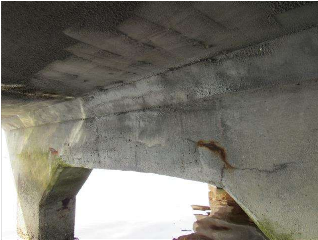
Bent 284 Cap 1: 6' OF LONGITUDINAL CRACKS UP TO 1/16", WITH RUST STAINING, AT RANDOM THROUGHOUT EAST AND WEST FACES.
