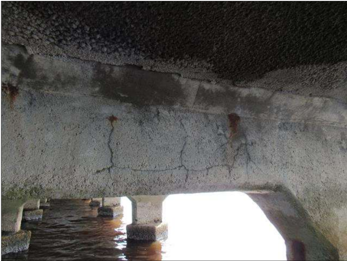
Bent 280 Cap 1: (PAR) 3' X 1' AREA OF UP TO 1/16" WIDE MAP CRACKING WITH RUST STAINING, WEST FACE, BAY 3.
