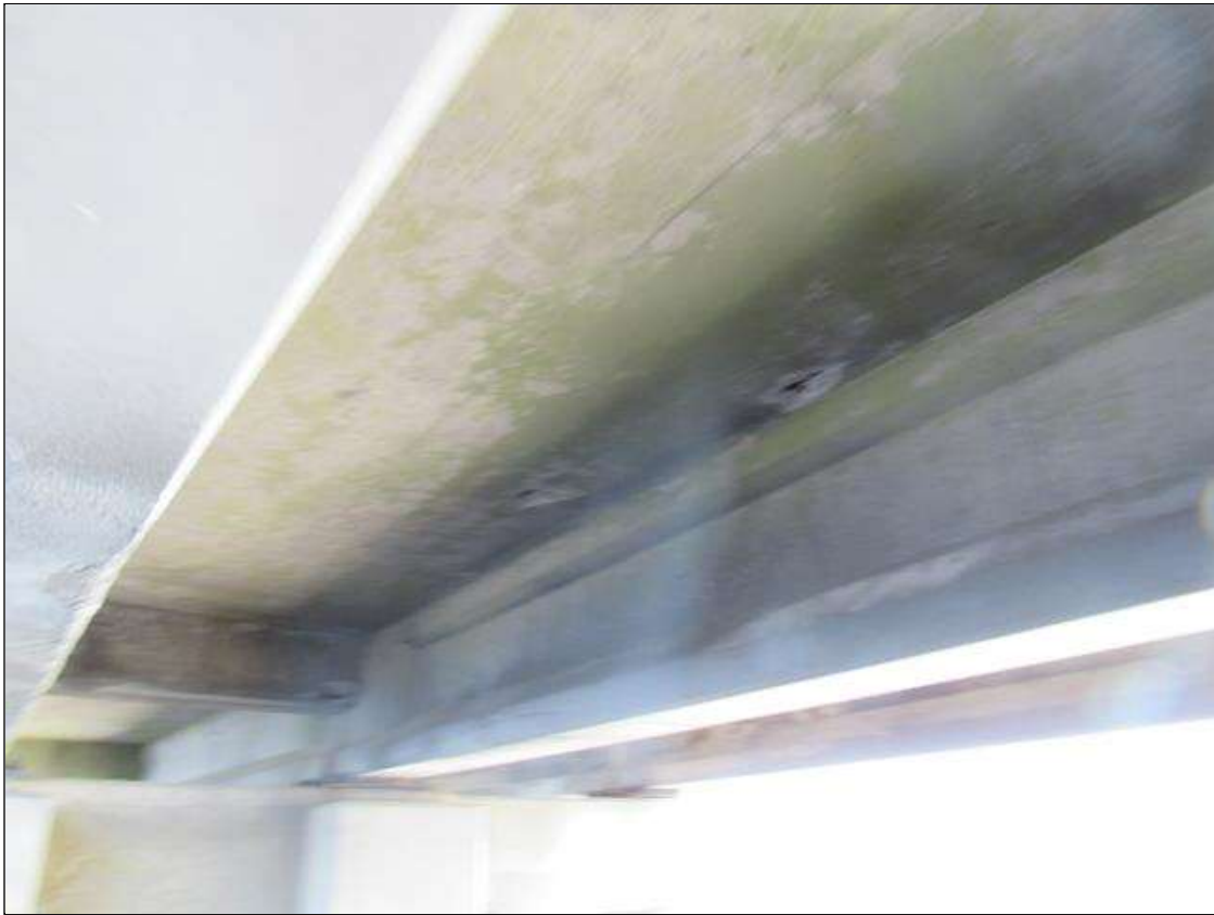
Span 5 Deck: (3) UP TO 14" X 10" X 1" SPALLS, WITH EXPOSED REINFORCING, DECK UNDERSIDE, BETWEEN BEAMS 2 AND 3, 10' FROM BENT 5.
