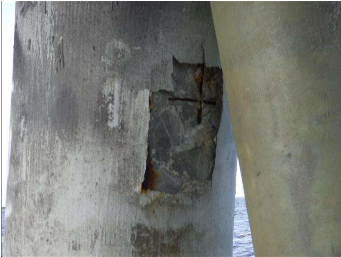
Bent 127 Pile 2: PILE HAS BEEN JACKETED, BEGINNING 1' FROM BOTTOM OF CAP, WITH PILE JACKET MISSING, AT RANDOM THROUGHOUT, EXTENDING BELOW WATERLINE, WITH 18" X 12" X 2" SPALL, WITH EXPOSED REBAR, EAST FACE, 5' FROM BOTTOM OF CAP.
