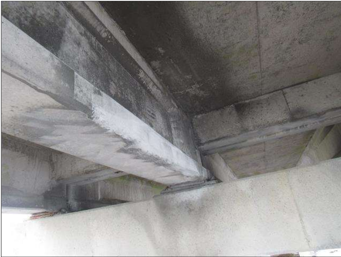
Span 33 Beam 3: 7' X UP TO 6" PATCHED AREA, BOTTOM FACE, EXTENDING 1' ONTO NORTH FACE, AT BENT 32.
