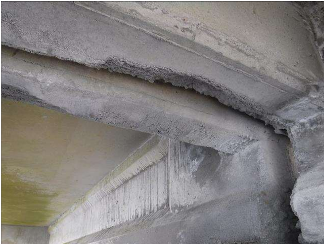
Span 112 Beam 1: 6' X UP TO 1.5' PATCHED AREA, 2" DEEP SPALL REMAINS, EAST FACE OF BENT 112 DIAPHRAGM, BETWEEN BEAMS 1 AND 2.
