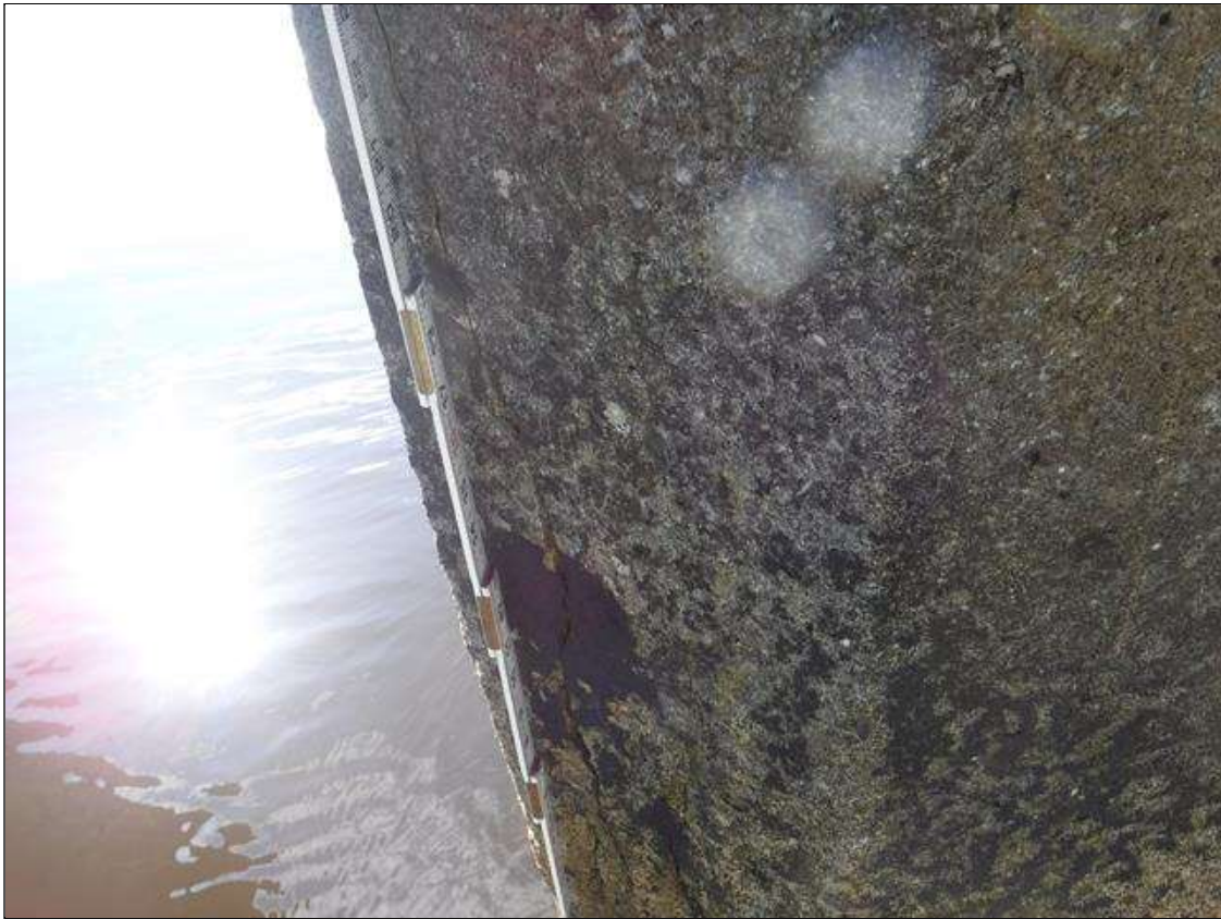
Bent 212 Pile 4: (PAR) 3' LONG HAIRLINE TO 1/8" CRACK, 8' BELOW CAP, DOWN 4' , MULTIPLE FACES. SCALING TO 1" DEEP WITH LOOSE AGGREGATE FROM WATERLINE TO MUDLINE.
