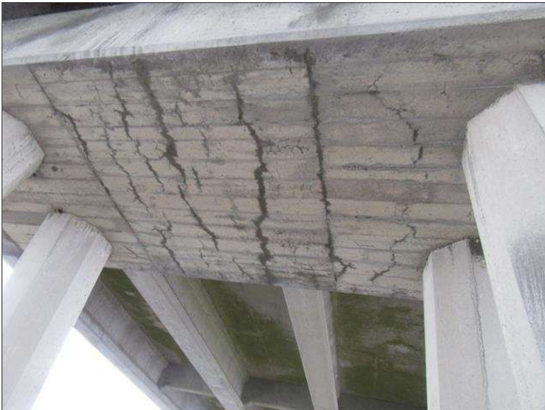
Bent 113 Cap 1: 15' X 5' AREA OF UP TO 1/32" TRANSVERSE CRACKS, BOTTOM FACE, BEGINNING 5' FROM NORTH END.
