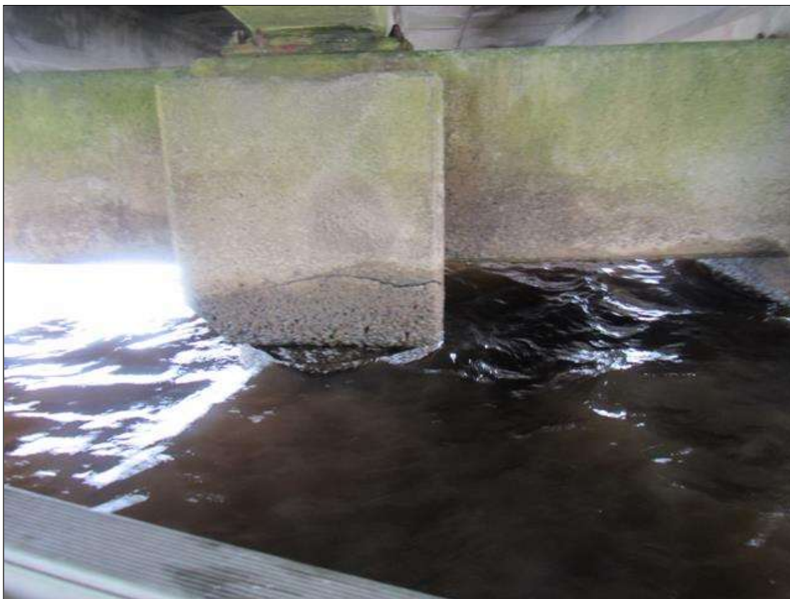
Bent 275 Cap 1: 3' X 8" DELAMINATION, WEST FACE, PILE 2 BLOCK-OUT.
