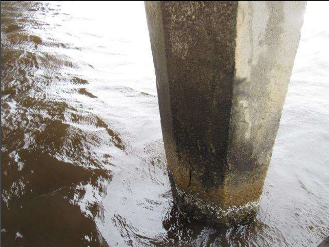
Bent 81 Pile 6: (PAR) 4' X 0.25" VERTICAL CRACK WITH SURROUNDING DELAMINATION ON NORTH FACE, BEGINNING 8' FROM BOTTOM OF CAP
