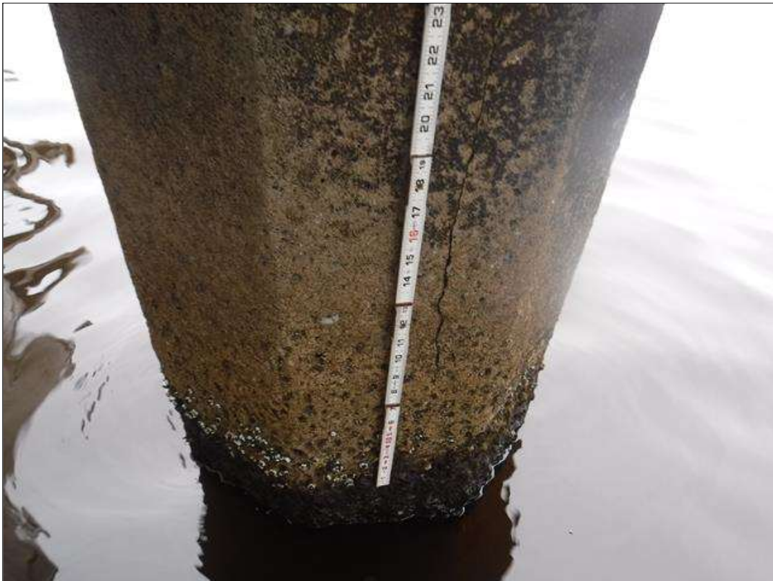
Bent 243 Pile 1: (PAR) 3' X 1/16" CRACKS WITH SURROUNDING DELAMINATION ON SOUTH FACE 7' FROM BOTTOM OF CAP
