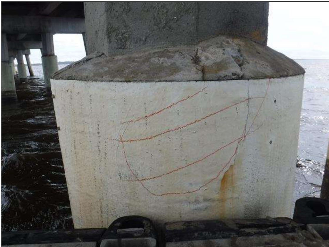
Bent 176 Pile 2: 12" X 5" DELAMINATION, WEST FACE ON TOP OF PILE JACKET, 5.25' FROM BOTTOM OF CAP.
