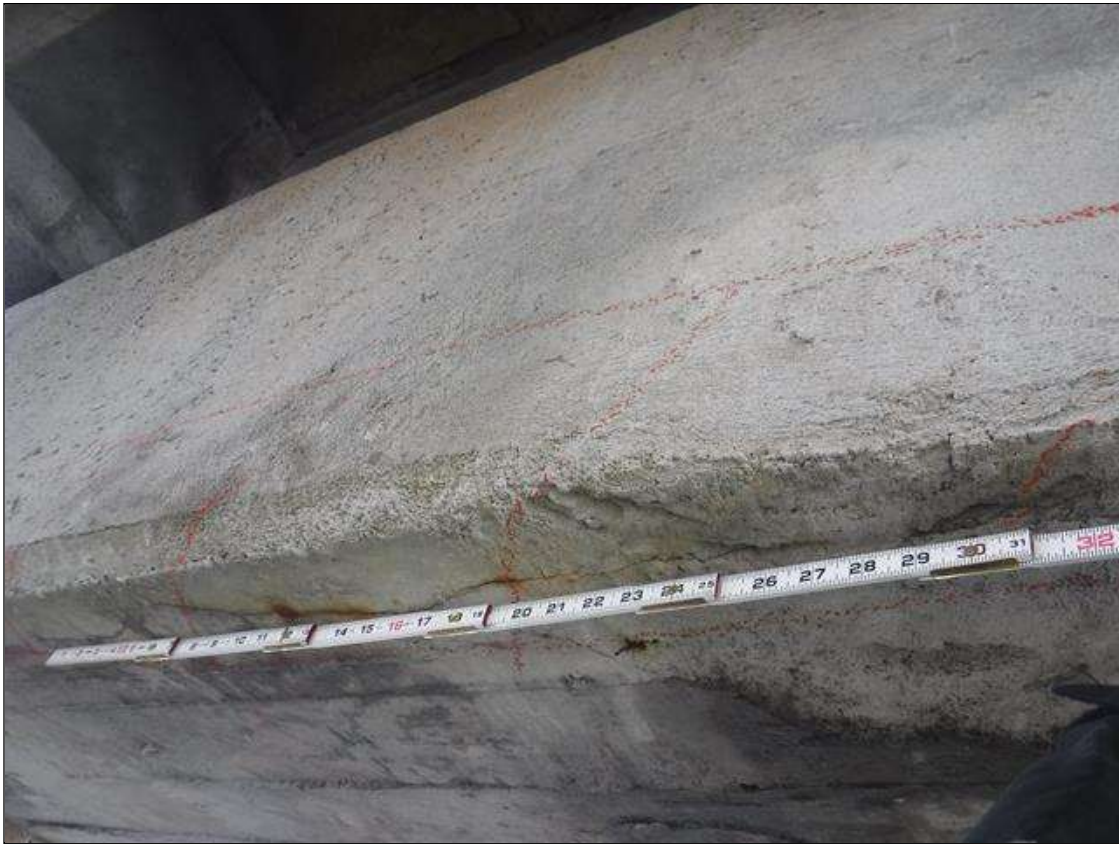
Bent 172 Cap 1: 40" X 6" HIGH X 6" DEEP DELAMINATION ON WEST BOTTOM CORNER BETWEEN BEAMS 1 AND 2
