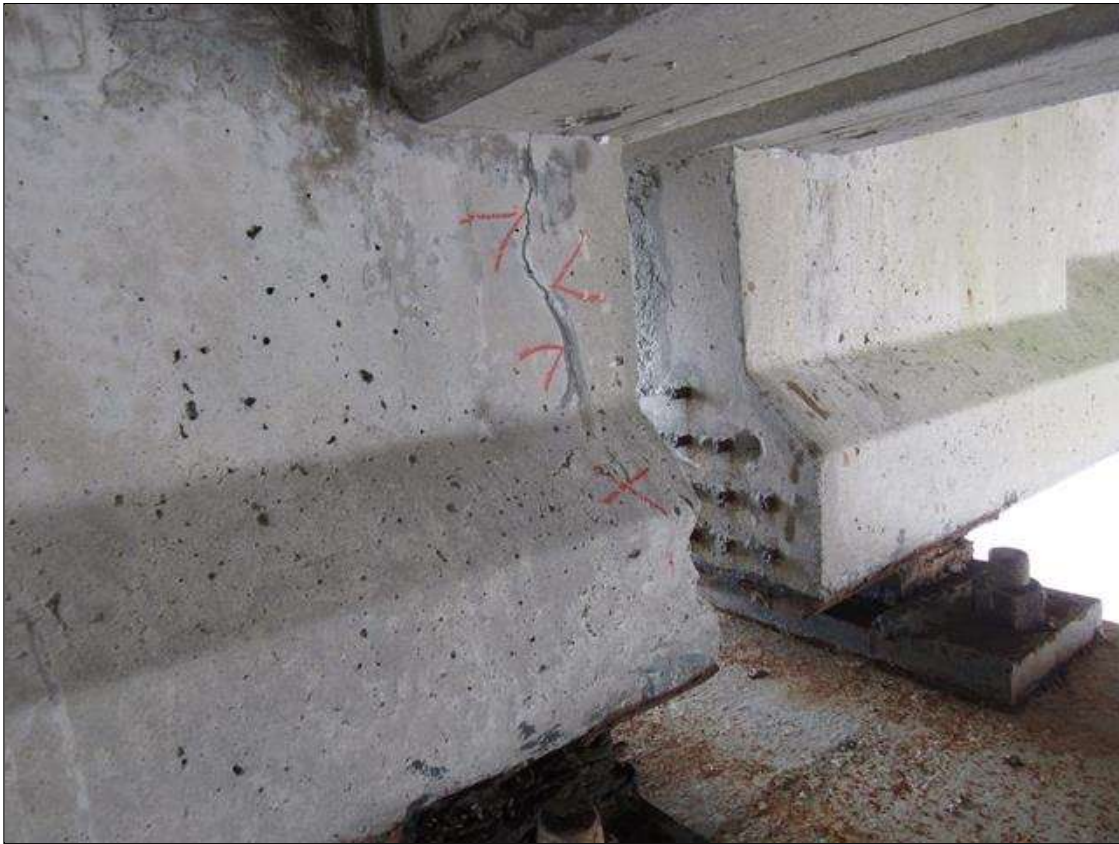
Span 41 Beam 1: (PAR) 11" LONG X UP TO 1/32" WIDE VERTICAL CRACK ON SOUTH FACE AT BENT 41
