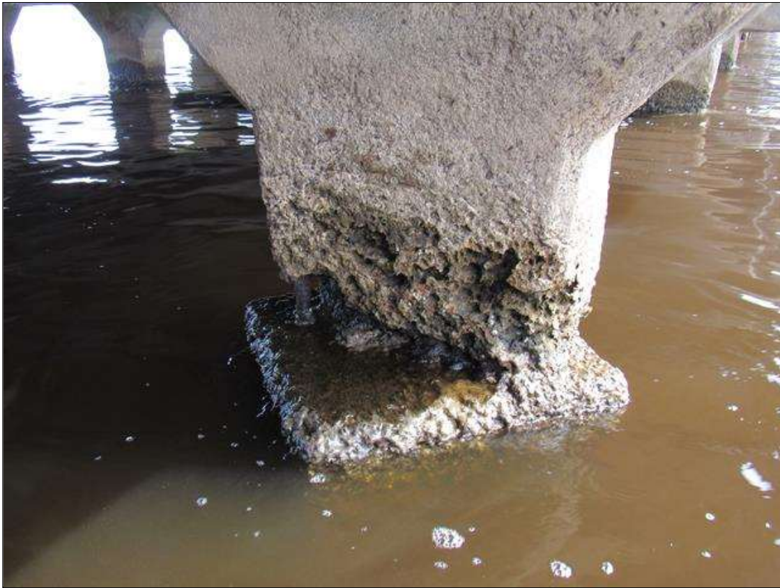
Bent 287 Pile 4: (PAR) 6" DEEP X 8" HIGH X FULL WIDTH SPALL WITH EXPOSED REBAR WITH 25% SECTION LOSS AROUND BASE OF COLUMN AND TOP OF FOOTING
