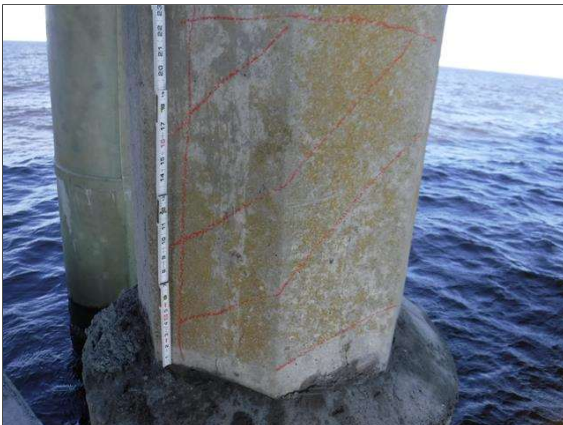
Bent 118 Pile 2: 2' X 2' DELAMINATION, SOUTH FACE, 6' FROM BOTTOM OF CAP.
