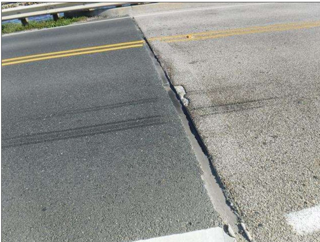
Span 1 Wearing Surface: 8" X 3" X 1/2" DEEP SPALL LOCATED IN RIGHT TRAVEL LANE
