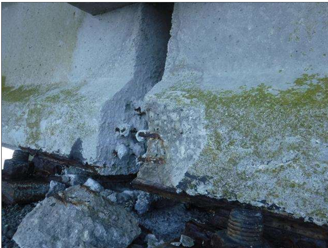
Span 141 Beam 1: (PAR) 6" X 6" X 2" DEEP SPALL WITH EXPOSED STRAND ON NORTH FACE AT BENT 141
