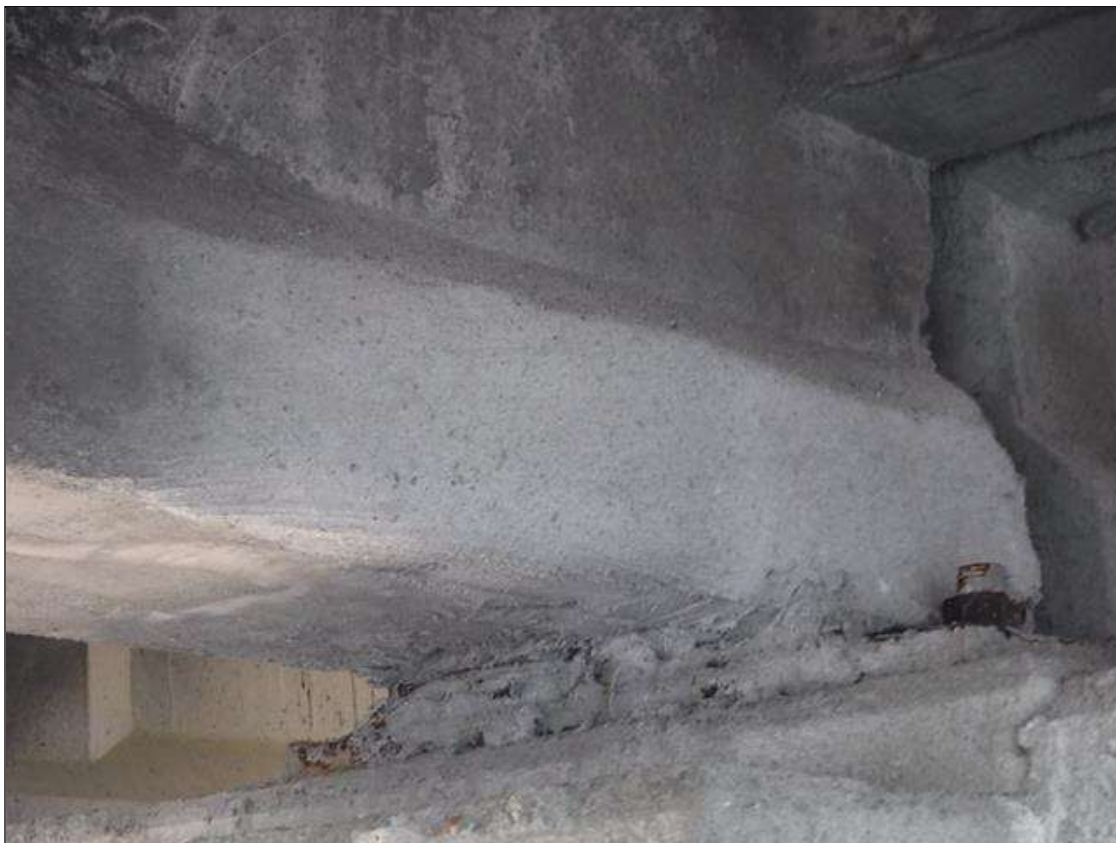
Span 30 Beam 2: 3' X 1' PATCHED AREA ON NORTH FACE AT BENT 29.
