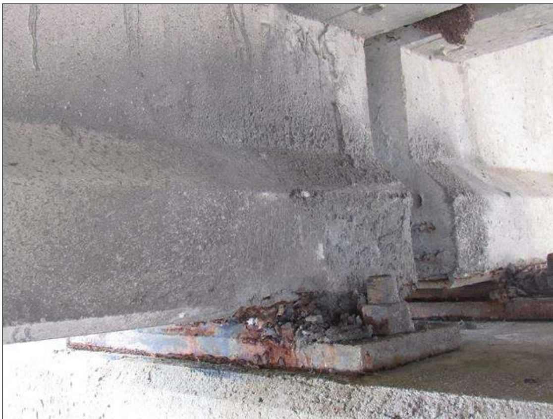
Span 44 Beam 1: 10" X 10" PATCHED AREA, SOUTH FACE, AT BENT 44.
