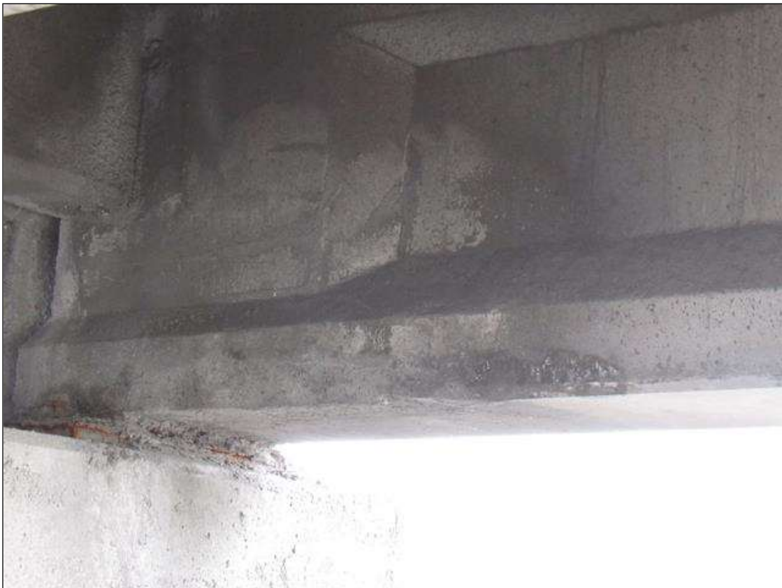
Span 33 Beam 1: 4' X UP TO 6" PATCHED AREA, BOTTOM FACE, EXTENDING 4" ONTO NORTH FACE, AT BENT 32.
