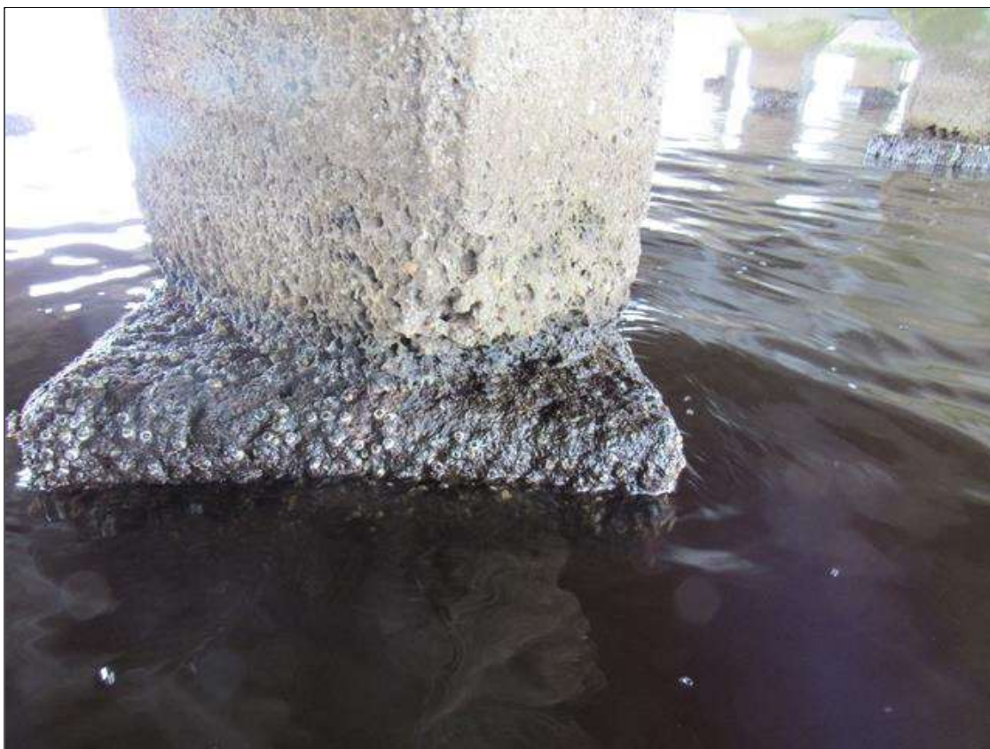
Bent 286 Pile 2: 12" X 2" X 2" DEEP SPALL WITH EXPOSED REINFORCING ON NORTH FACE LOCATED AT BOTTOM OF PILE 2
