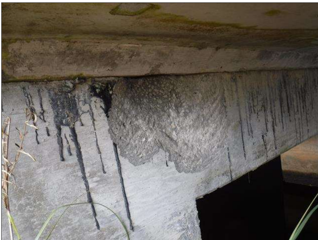
Bent 325 Cap 1: 24" X 24" X 2" SPALL, EAST FACE, ABOVE PILE 4.
