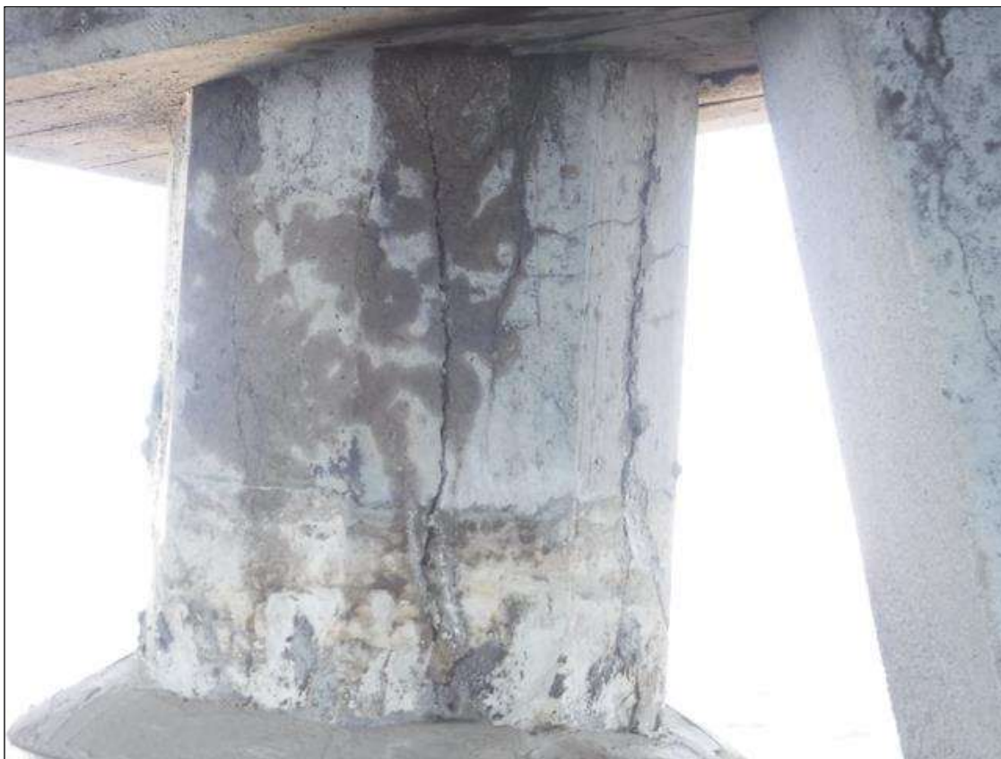
Bent 13 Saved Pile 5: (PAR) 3' X 1' DELAMINATION, WEST FACE, BEGINNING AT BOTTOM OF CAP TO TOP OF PILE JACKET
