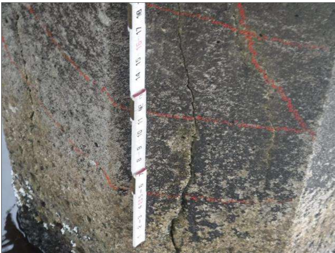
Bent 242 Pile 1: (PAR) 48" X 1" DELAMINATION, SOUTH FACE, 6' FROM BOTTOM OF CAP.
