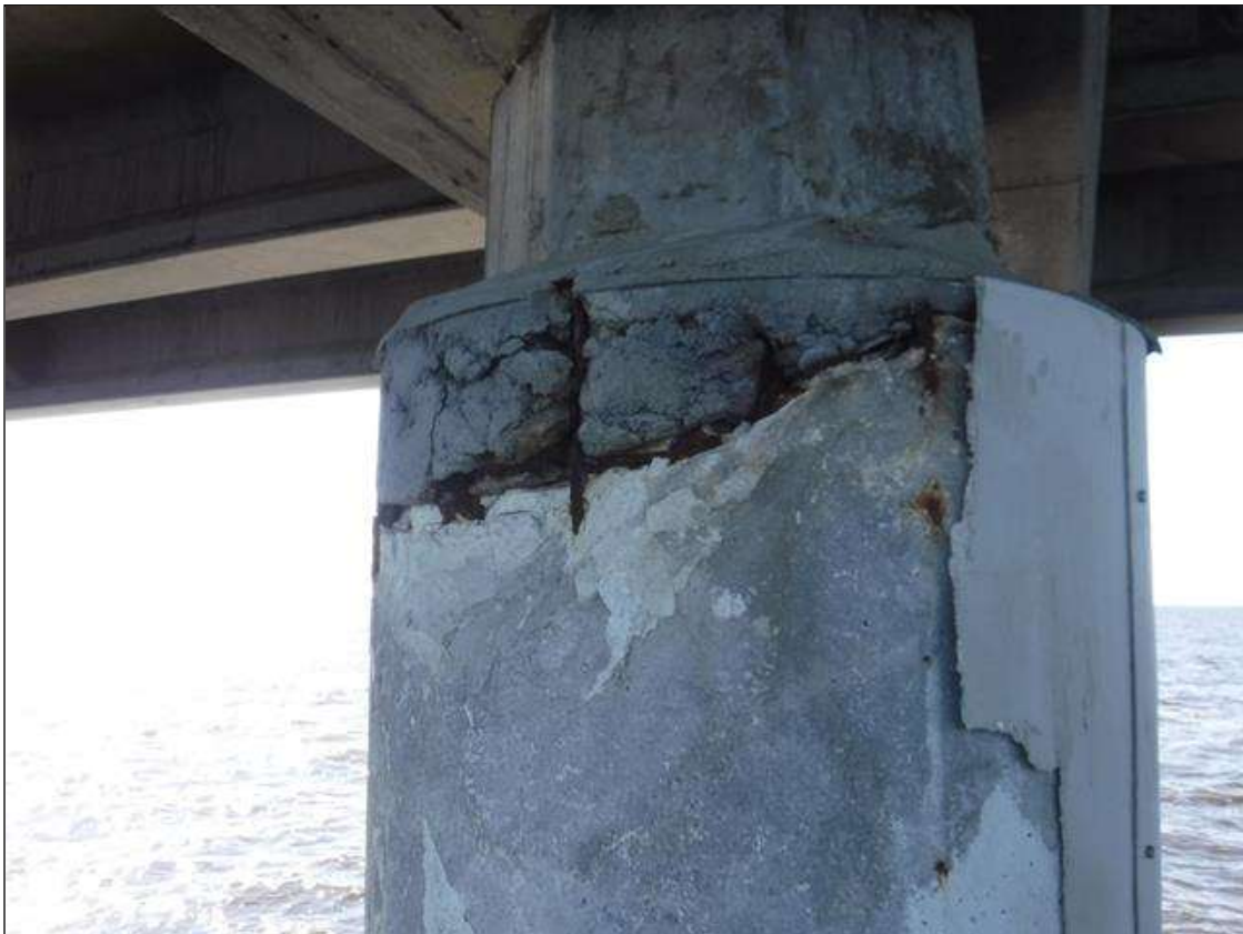
Bent 15 Saved Pile 2: (PAR) 6" X 12" X UP TO 1/2" SPALL WITH EXPOSED REBAR, REBAR HAS 50% SECTION LOSS, NORTH FACE, 2' FROM BOTTOM OF CAP.
