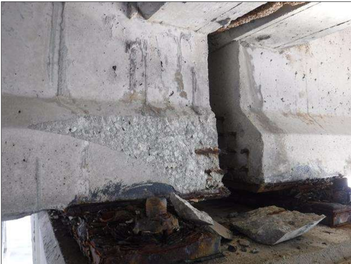
Span 79 Beam 3: (PAR) 15" X 8" X 2" DEEP SPALL WITH EXPOSED STRANDS ON SOUTH FACE AT BENT 79
