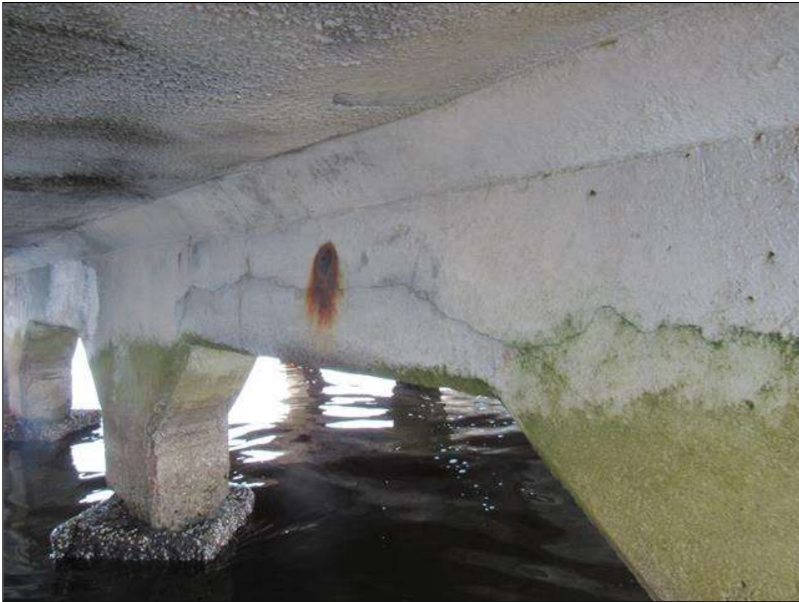
Bent 285 Cap 1: (PAR) 9' OF UP TO 1/16" TRANSVERSE AND LONGITUDINAL CRACKS WITH RUST STAINING, AT RANDOM THROUGHOUT EAST AND WEST FACES.
