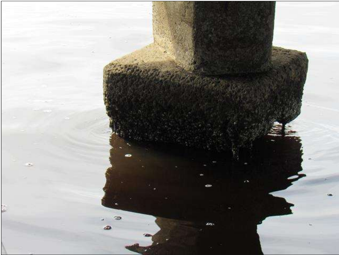
Bent 280 Pile 4: (PAR) 8' X 1' X 8" DEEP SPALL WITH EXPOSED REINFORCING LOCATED ON ALL FACES
