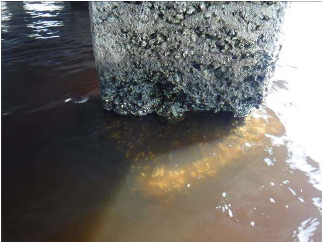
Bent 297 Pile 4: (PAR) 12" X 20" X 6" SPALL, WITH EXPOSED REBAR ON NORTH FACE, 2' FROM BOTTOM OF CAP. REBAR HAS UP TO COMPLETE SECTION LOSS
