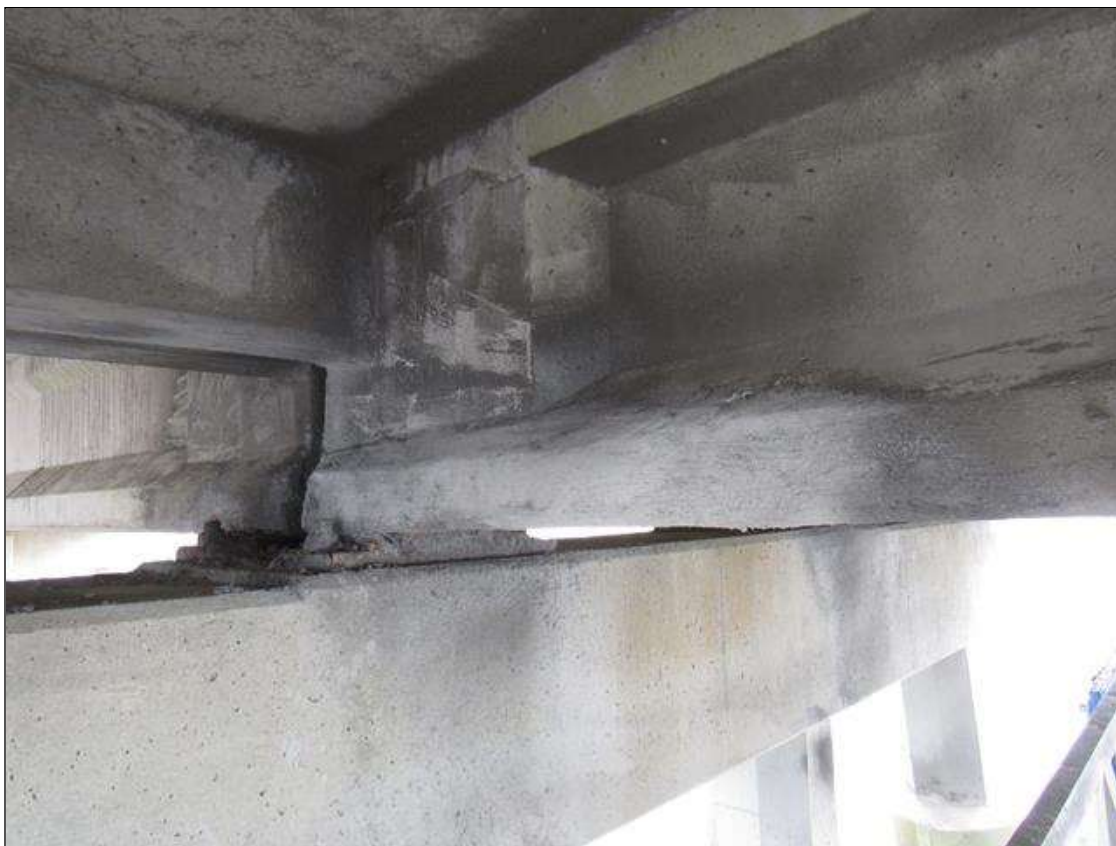
Span 60 Beam 2: (2) UP TO 55" X 12" X 6" CORNER PATCHED AREAS, NORTH AND SOUTH FACES, AT BENT 60.
