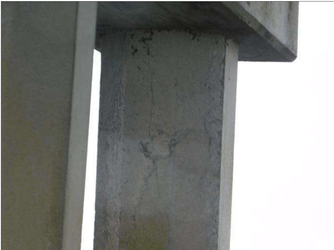
Bent 91 Saved Pile 1: (PAR) (2) UP TO 3' X 0.014" VERTICAL CRACKS, SOUTH FACE, BEGINNING AT BOTTOM OF CAP, WITH ADJACENT 3' X UP TO 1' DELAMINATION.
