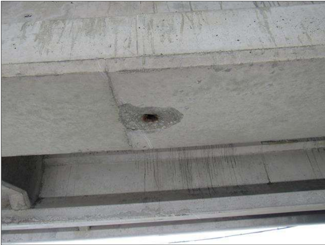
Span 59 Beam 3: 7" X 5" X UP TO 1" SPALL, WITH EXPOSED REINFORCING, BOTTOM FACE, 5' EAST OF MID SPAN.
