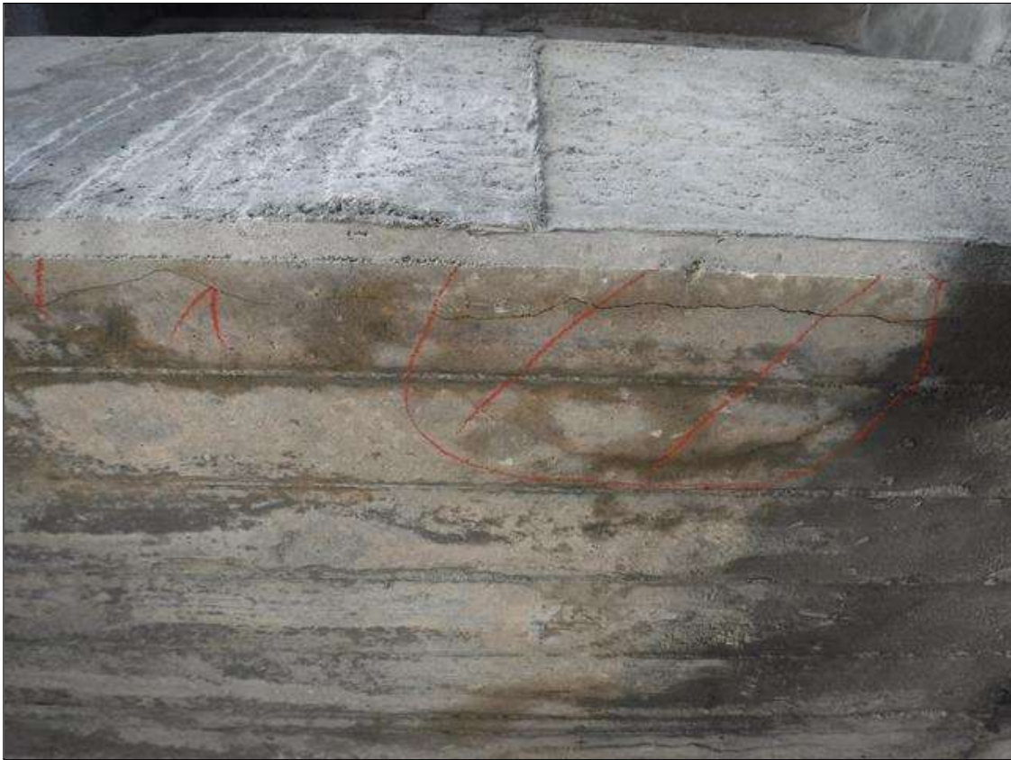
Bent 170 Cap 1: 2' DIAMETER DELAMINATION WITH 3' LONG HAIRLINE CRACK IN BOTTOM OF CAP BETWEEN PILES 2 AND 3
