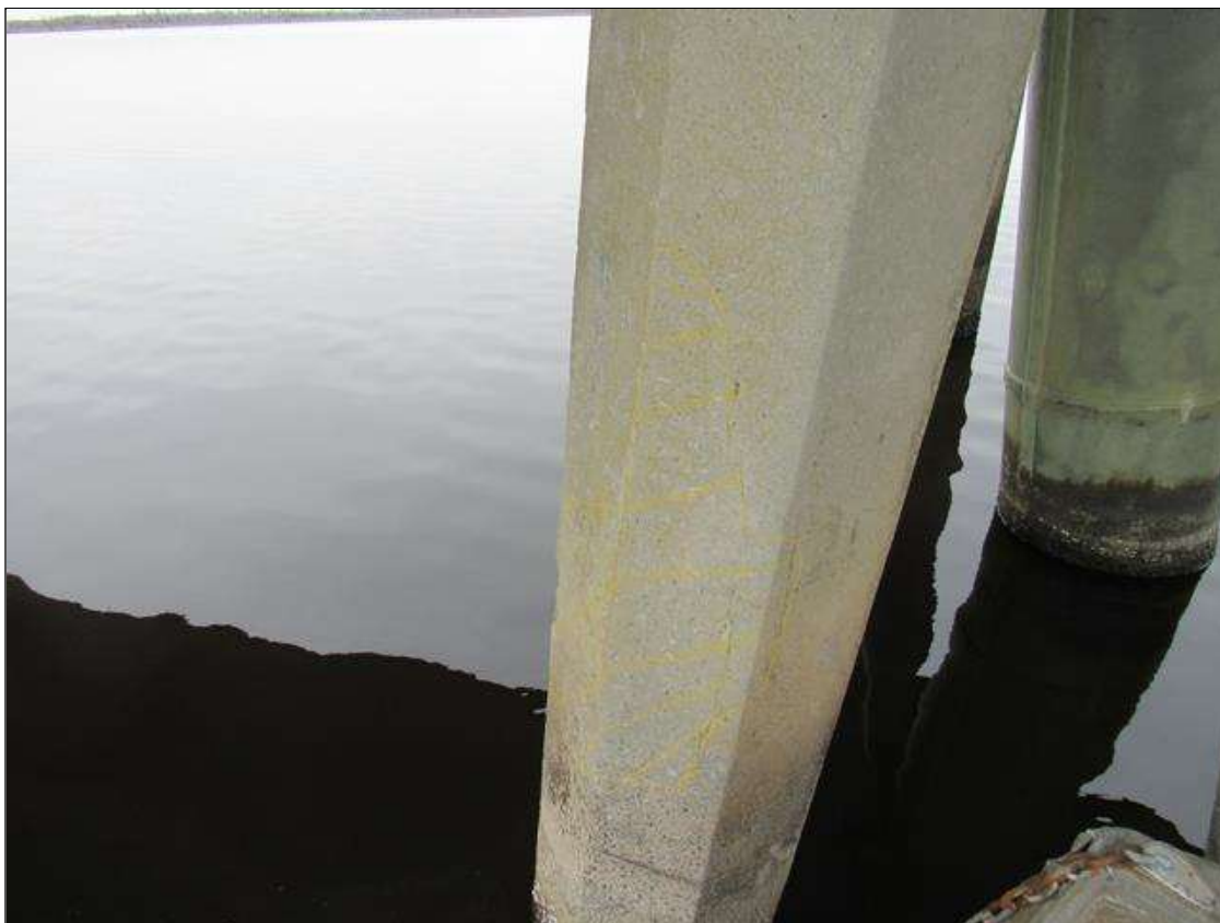
Bent 37 Saved Pile 4: 5' X 18" DELAMINATION, SOUTH FACE, 5' FROM BOTTOM OF CAP.
