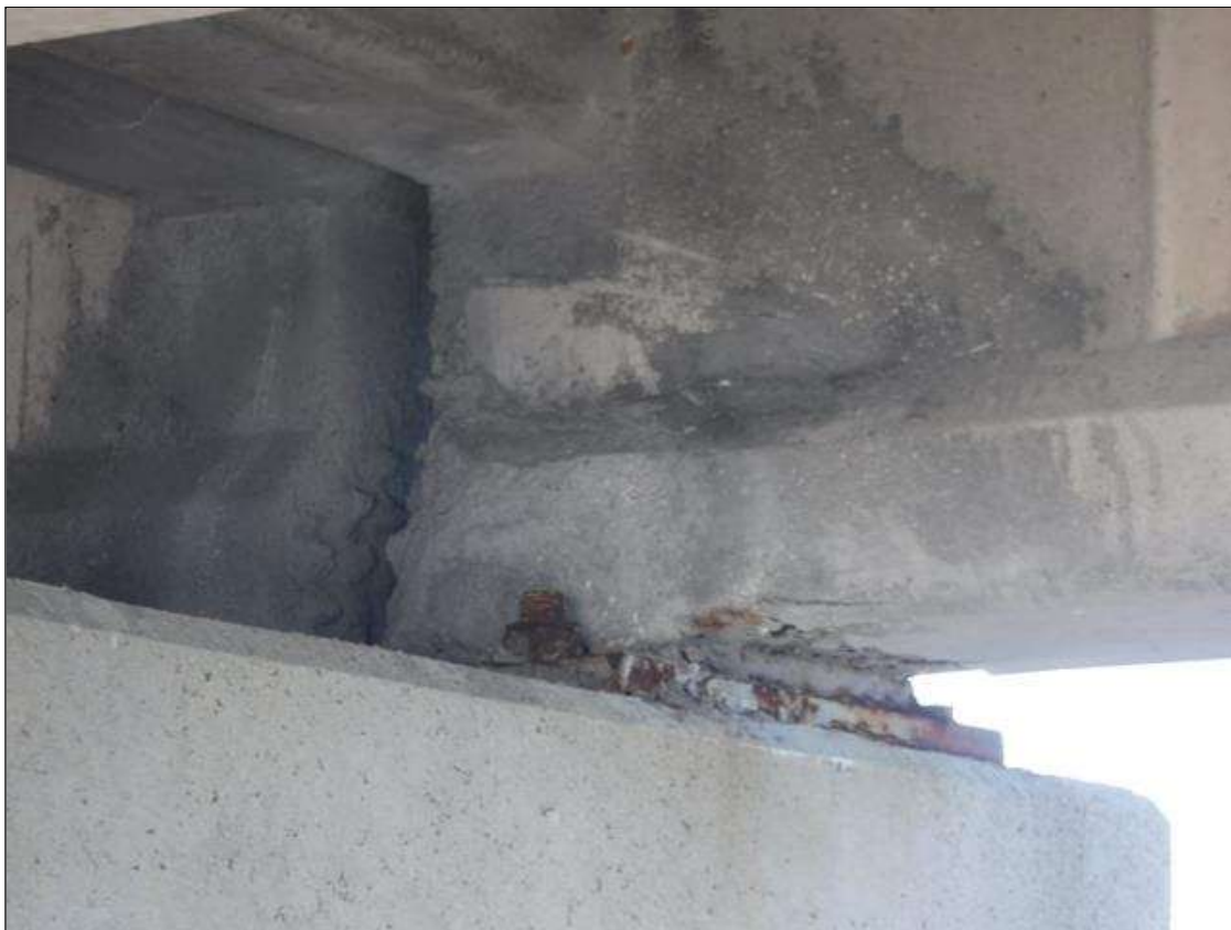
Span 23 Beam 1: 16" LONG X 10" TALL PATCHED AREA ON SOUTH FACE AT BENT 22.
