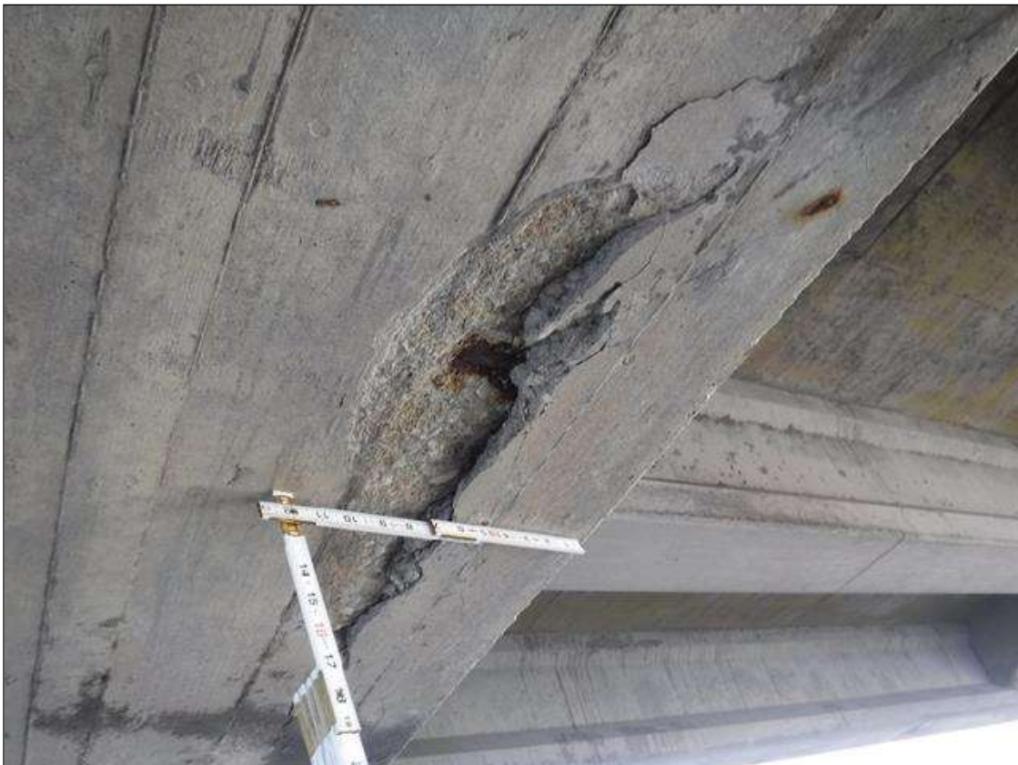
Bent 217 Cap 1: 24" X UP TO 6" X 1" SPALL WITH EXPOSED REINFORCING, BOTTOM OF CAP, BETWEEN PILES 2 AND 3.
