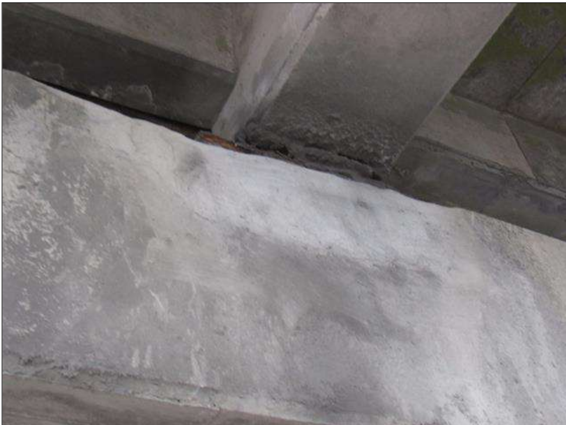
Bent 55 Cap 1: 48" X 12" FAILED PATCHED AREA, EAST FACE, BENEATH BEAM 3.
