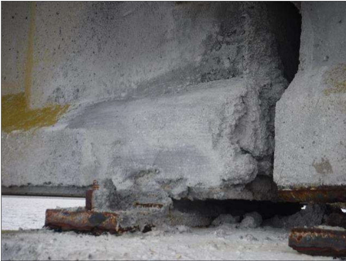
Span 188 Beam 1: 12" X 12" PATCHED AREA, NORTH FACE, AT BENT 187.
