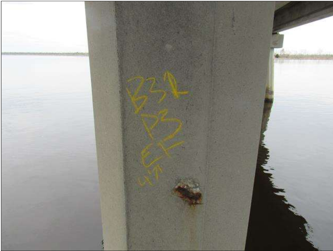
Bent 32 Saved Pile 3: 3" DIAMETER X 1/4" DEEP SPALL ON EAST FACE LOCATED 3' FROM BOTTOM OF CAP
