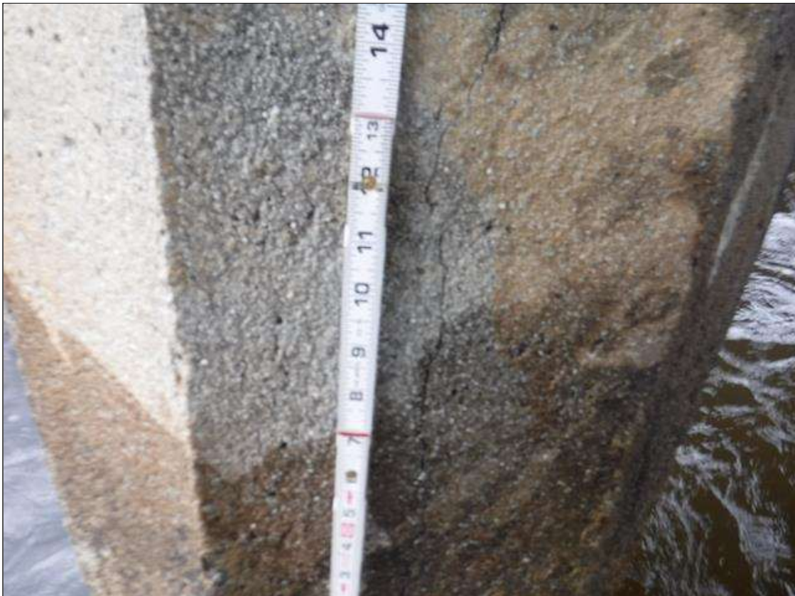
Bent 192 Pile 4: (PAR) HAIRLINE TO 1/8" CRACKS, 8' BELOW CAP, DOWN 4', MULTIPLE FACES. SCALING TO 1" DEEP WITH LOOSE AGGREGATE FROM WATERLINE TO MUDLINE.
