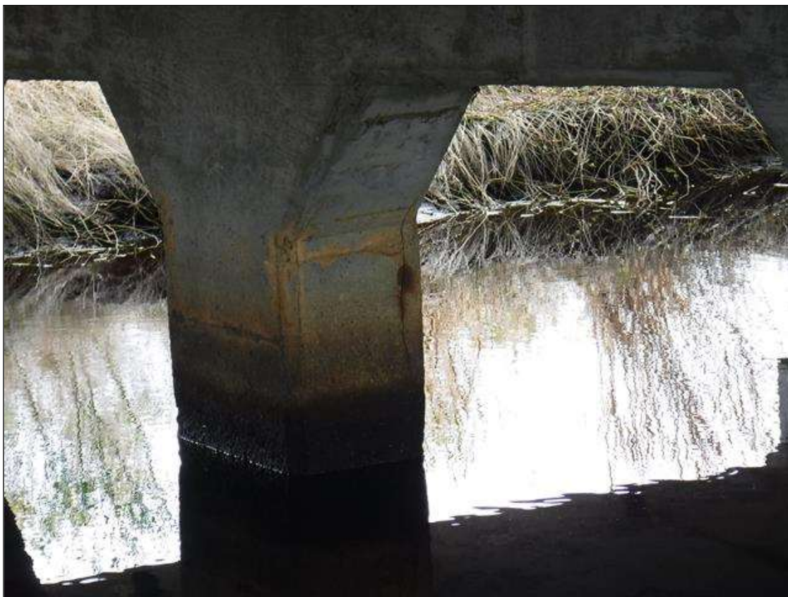
Bent 323 Pile 2: (2) UP TO 18" X 3" DELAMINATIONS, NORTH AND SOUTH FACES, AT BOTTOM OF CAP.
