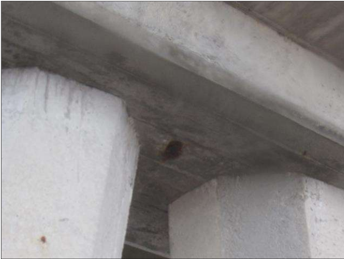
Bent 61 Cap 1: 4" DIAMETER X 1/2" DEEP SPALL WITH EXPOSED REBAR ON BOTTOM FACE BETWEEN PILES 4 AND 5
