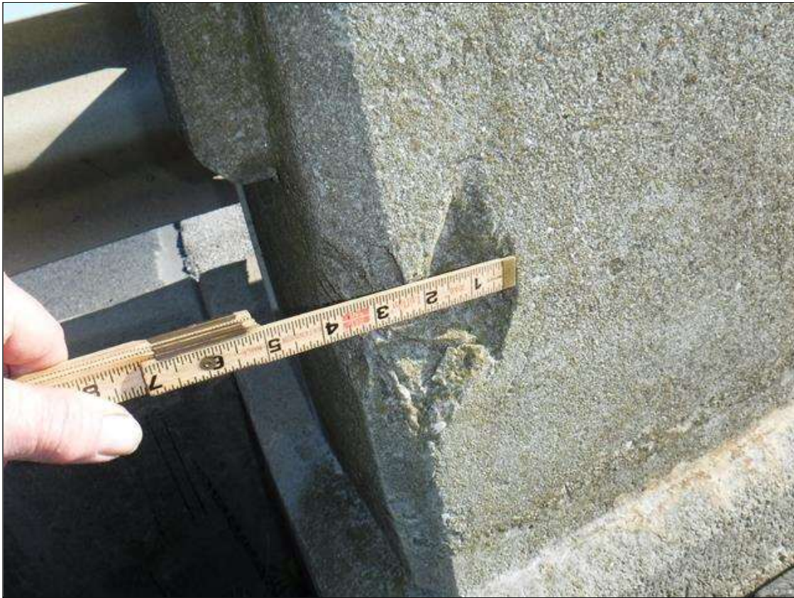
Span 1 Right Bridge Rail: 3 1/2" X 5" X 2" SPALL ON RIGHT FACE LOCATED AT NEAR RIGHT END POST
