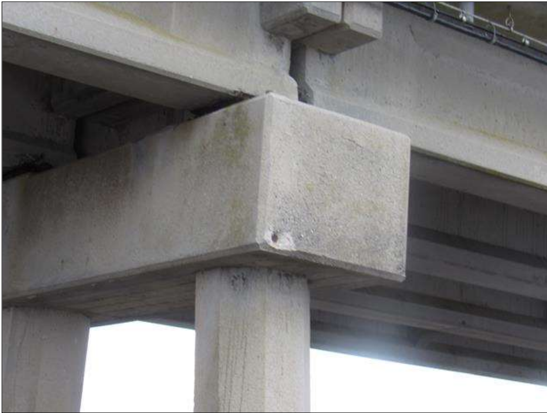
Bent 99 Cap 1: 6" X 5" X 1" DEEP SPALL WITH EXPOSED REINFORCEMENT ON SOUTH END OF CAP
