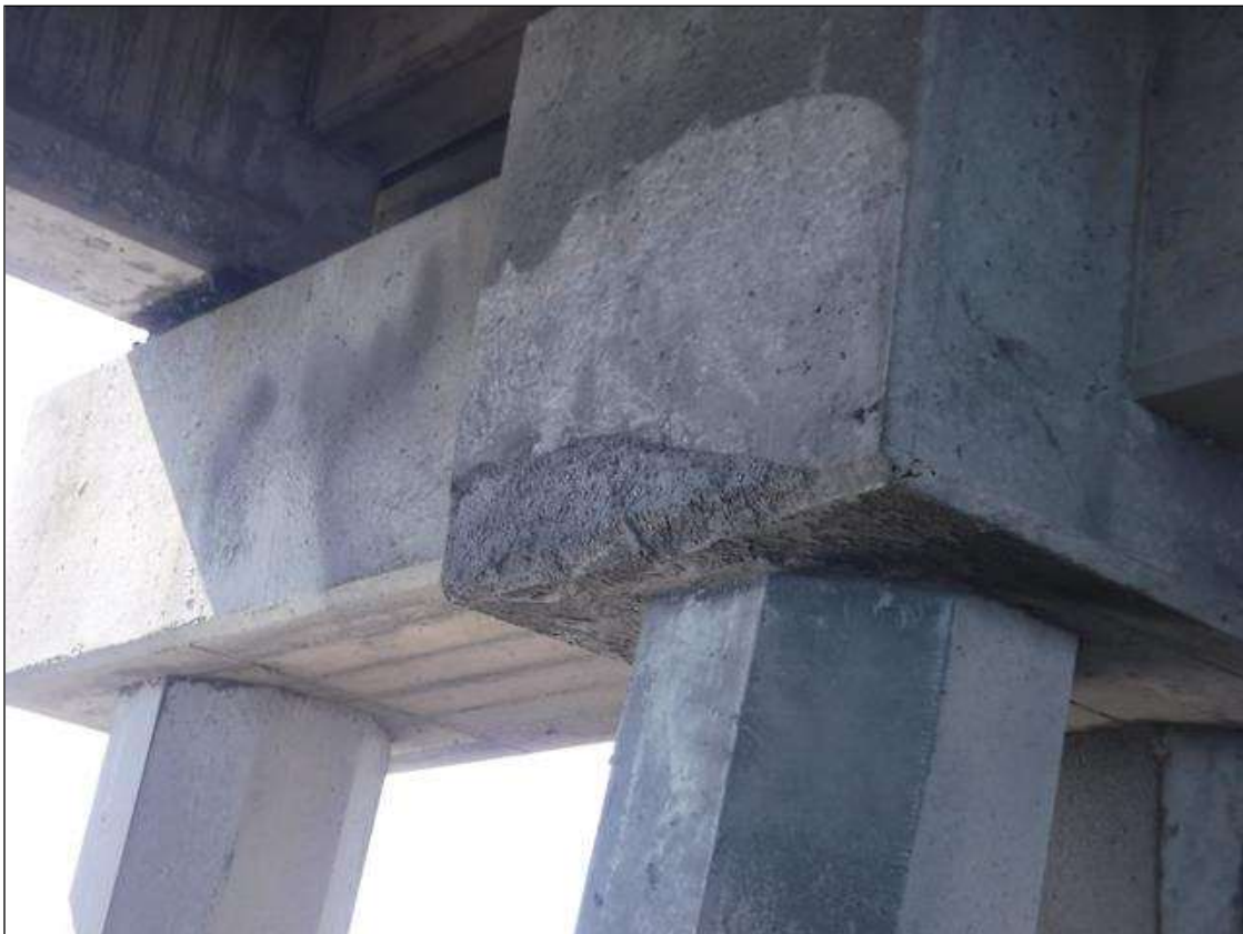
Bent 25 Cap 1: 24" X 12" PATCHED AREA IN EAST FACE ABOVE PILE 5
