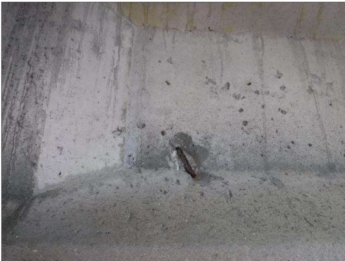
Span 128 Beam 4: (PAR) 2" DIAMETER X 1/2" SPALL, WITH EXPOSED STRAND, NORTH FACE, 3' FROM BENT 128.
