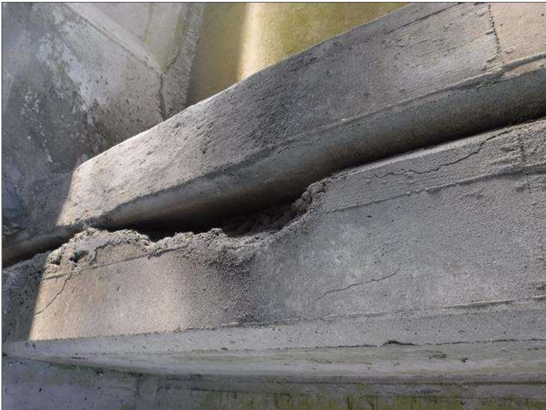
Span 122 Beam 4: 2' X 3" X 3" DEEP SPALL WITH EXPOSED REBAR ON EAST FACE OF BAY 3 DIAPHRAGM AT BENT 122
