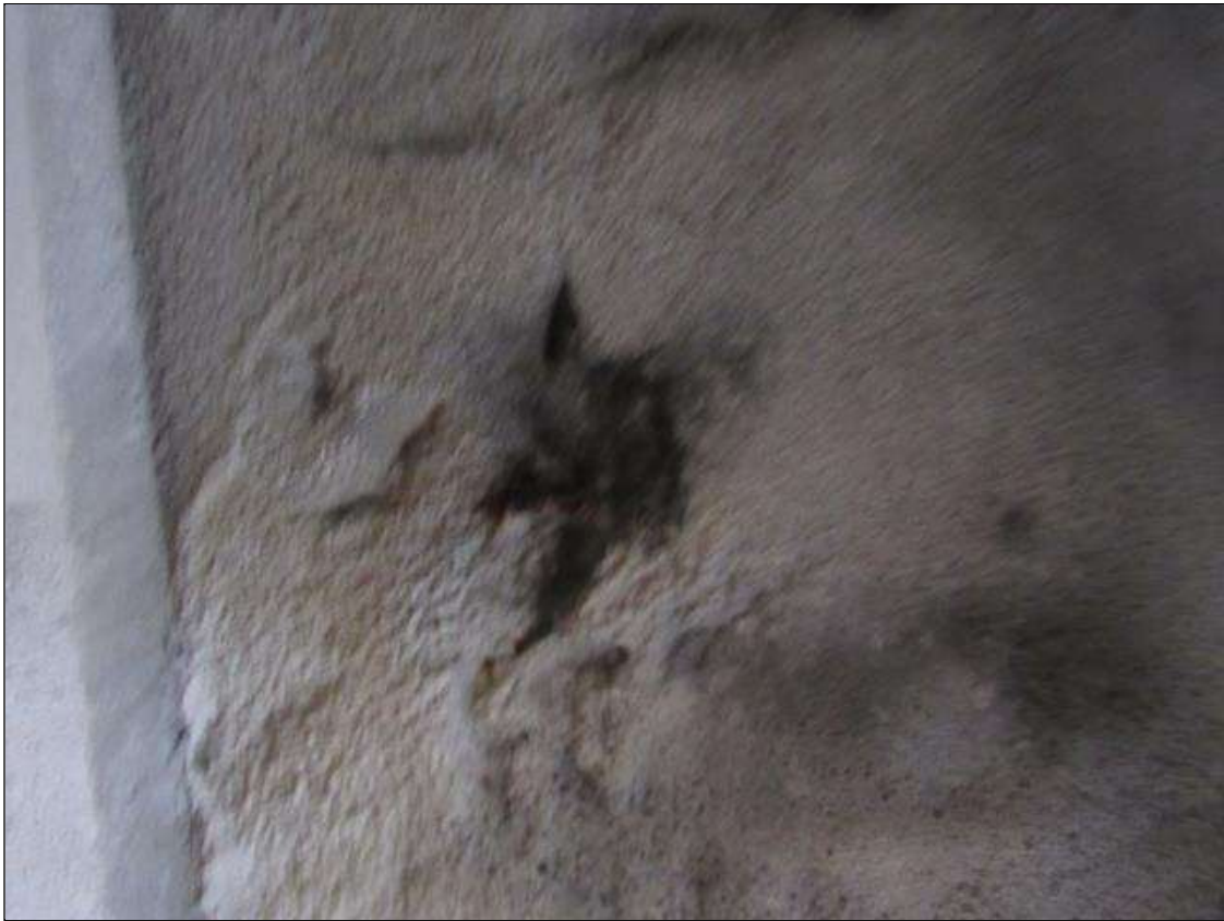
Span 1 Deck: 12" DIAPHRAGM FAILED PATCHED AREA ON UNDERSIDE OF DECK LOCATED 4' FROM END BENT 1 IN BAY 2
