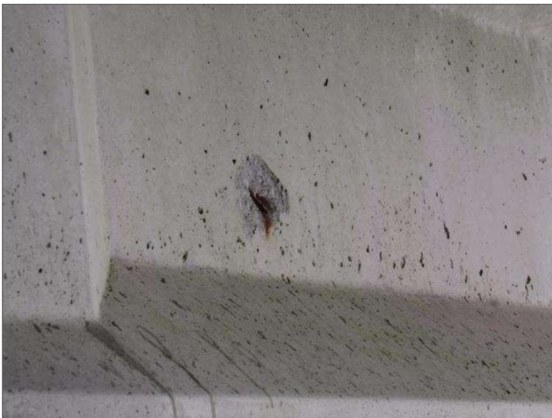
Span 46 Beam 1: 3" DIAMETER SPALL IN WEB, 5' FROM BENT 45.
