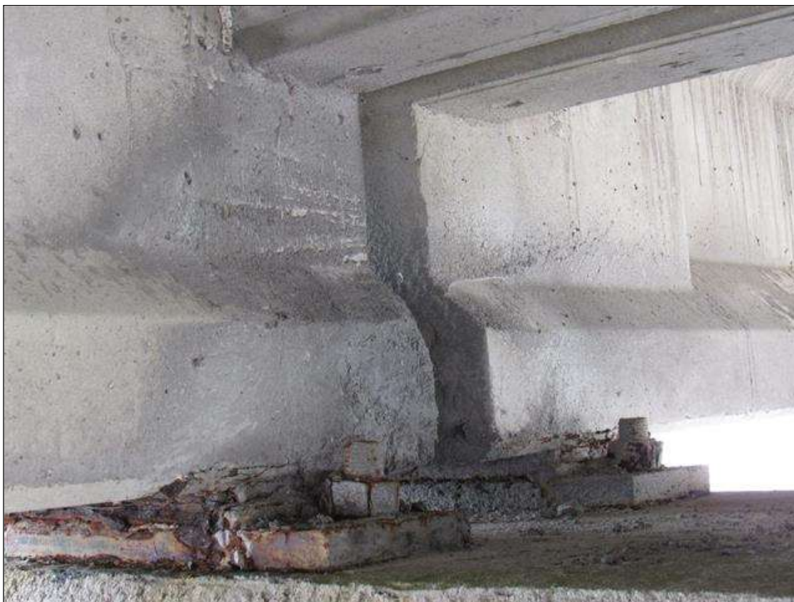
Span 50 Beam 1: 12" X 12" PATCHED AREA, SOUTH FACE, AT BENT 50.
