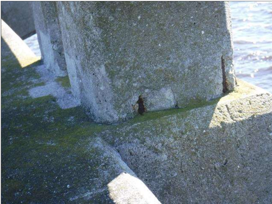
Span 54 Right Bridge Rail: (2) 3" X 3" X 3 1/4" SPALL WITH EXPOSED REBAR AT BOTTOM RIGHT CORNER LOCATED AT POST 3 FROM BENT 53
