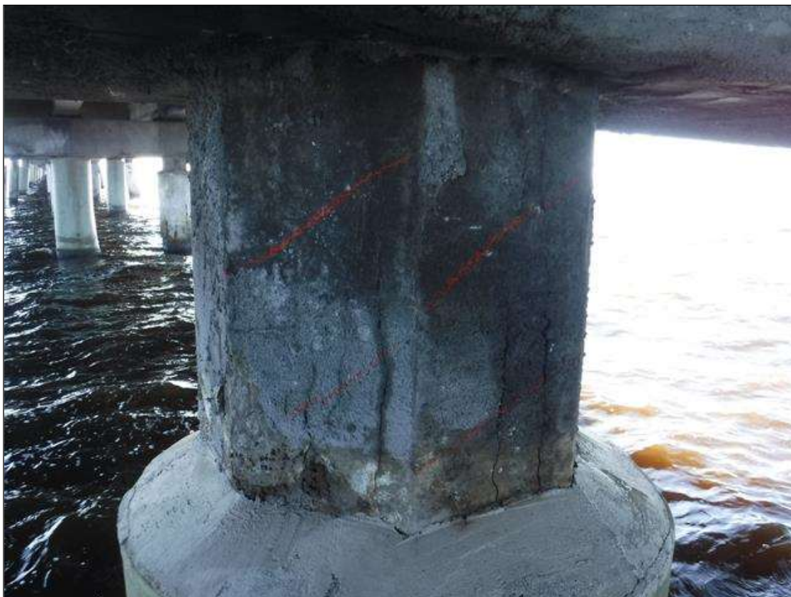
Bent 10 Saved Pile 2: 2' X 3' DELAMINATION, WEST FACE, BEGINNING AT TOP OF PILE.
