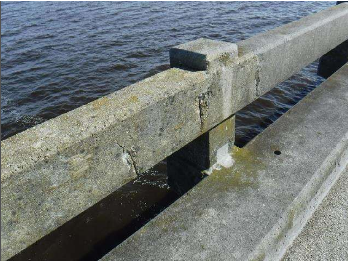
Span 150 Left Bridge Rail: (3) UP TO 8" X 4" X 1/2" SPALLS WITH EXPOSED REBAR ON RIGHT FACE LOCATED ON RAIL AT POST 5
