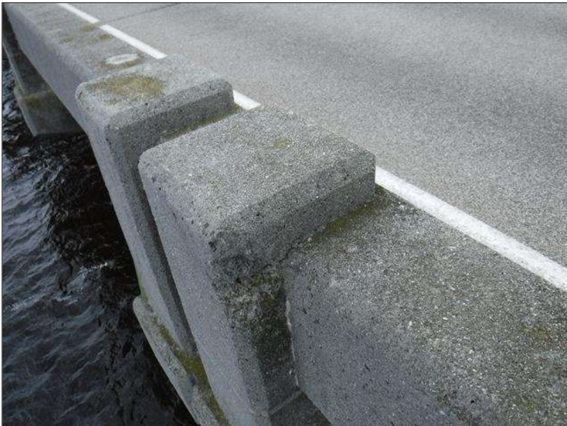
Span 191 Left Bridge Rail: 6" X 3" X 2" SPALL AT TOP LEFT CORNER LOCATED ON POST 6
