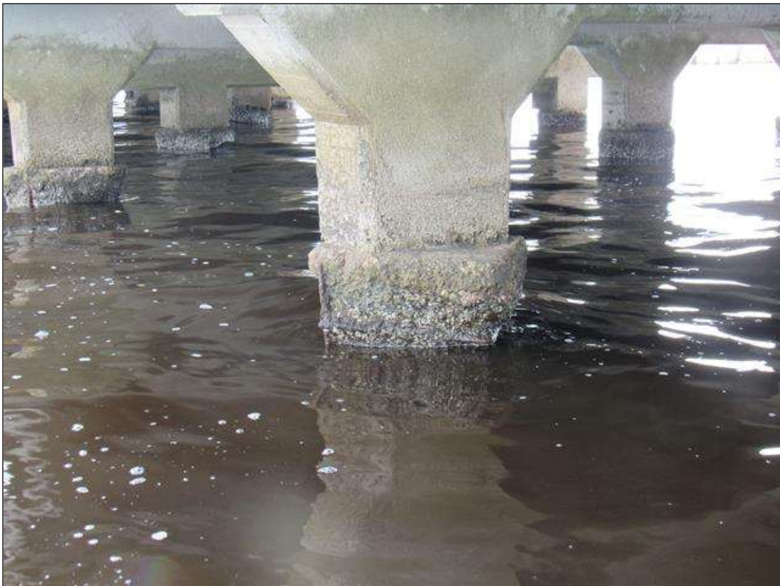
Bent 281 Pile 1: (PAR) 18" X 24" X 24" SPALL, WITH EXPOSED REINFORCING AND COMPLETE SECTION LOSS TO VERTICAL BARS, WEST FACE OF COLUMN FOOTING.
