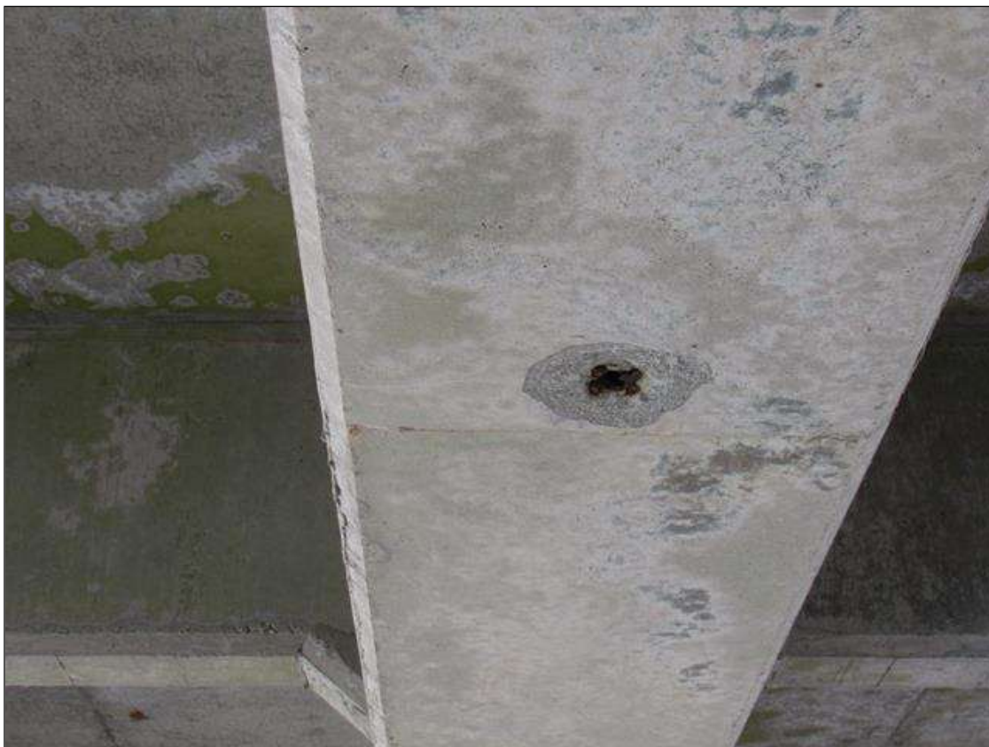
Span 63 Beam 3: 5" DIAMETER X UP TO 1/2" SPALL, WITH EXPOSED REINFORCING, BOTTOM FACE, 5' EAST OF MID SPAN.
