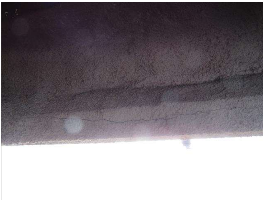
Span 2 Beam 4: (PAR) 16' X UP TO 0.25" LONGITUDINAL CRACK, BOTTOM FACE, BEGINNING AT BENT 2.
