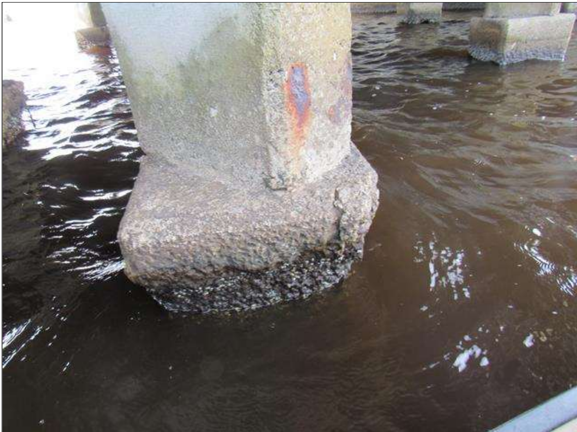
Bent 280 Pile 1: (PAR) 24" X 24" X 24" SPALL, WITH EXPOSED REBAR WITH COMPLETE SECTION LOSS, NORTH FACE OF COLUMN FOOTING.
