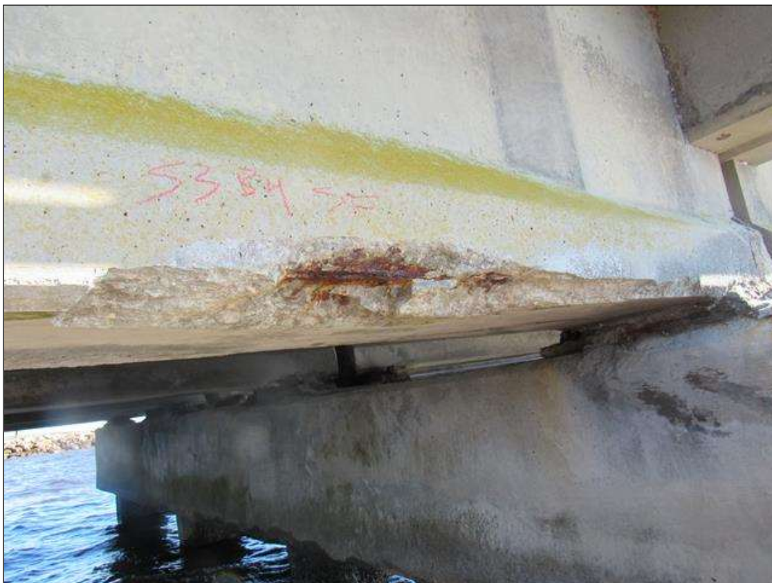
Span 3 Beam 4: (PAR) 48" X 8" X 2" SPALL, WITH EXPOSED STRAND, BOTTOM FACE, 3' FROM BENT 3.
