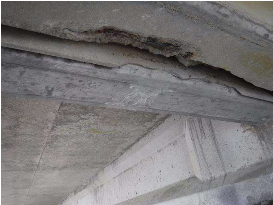
Span 107 Beam 2: (PAR) 4' X UP TO 6" X 6" SPALL, WITH EXPOSED REINFORCING, END DIAPHRAGM, BETWEEN BEAMS 2 AND 3, AT BENT 107.
