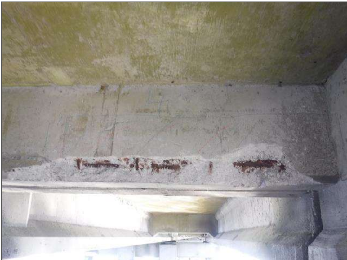
Span 134 Beam 3: (PAR) 5' X 10" X 3" DEEP SPALL WITH EXPOSED REBAR AND 4' X 1' SURROUNDING DELAMINATION ON WEST FACE BAY 3 DIAPHRAGM AT BENT 134
