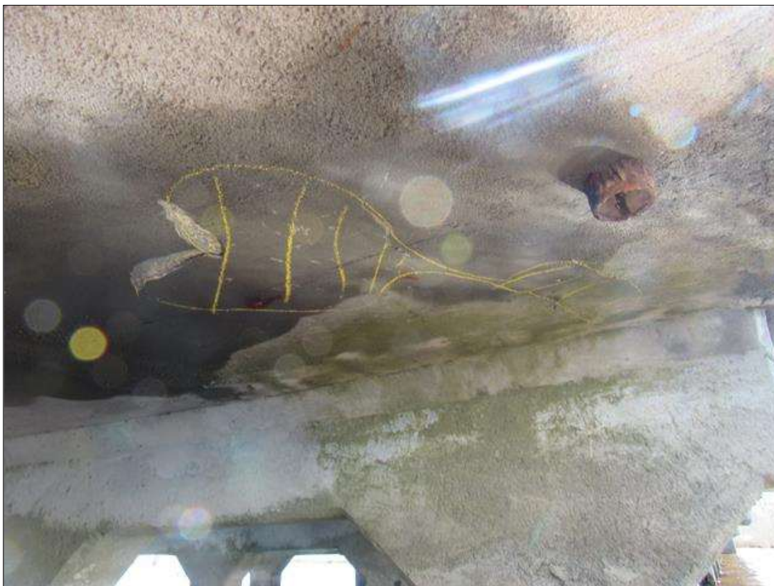
Span 285 Deck: 5 SF OF DELAMINATIONS, AT RANDOM THROUGHOUT DECK UNDERSIDE.
