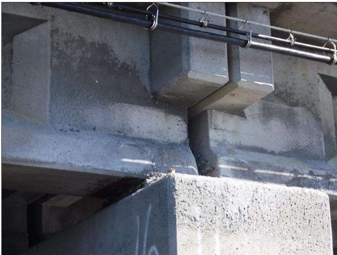
Span 16 Beam 4: 16" TALL X 12" LONG PATCHED AREA AT BENT 16 ON EXTERIOR SIDE.
