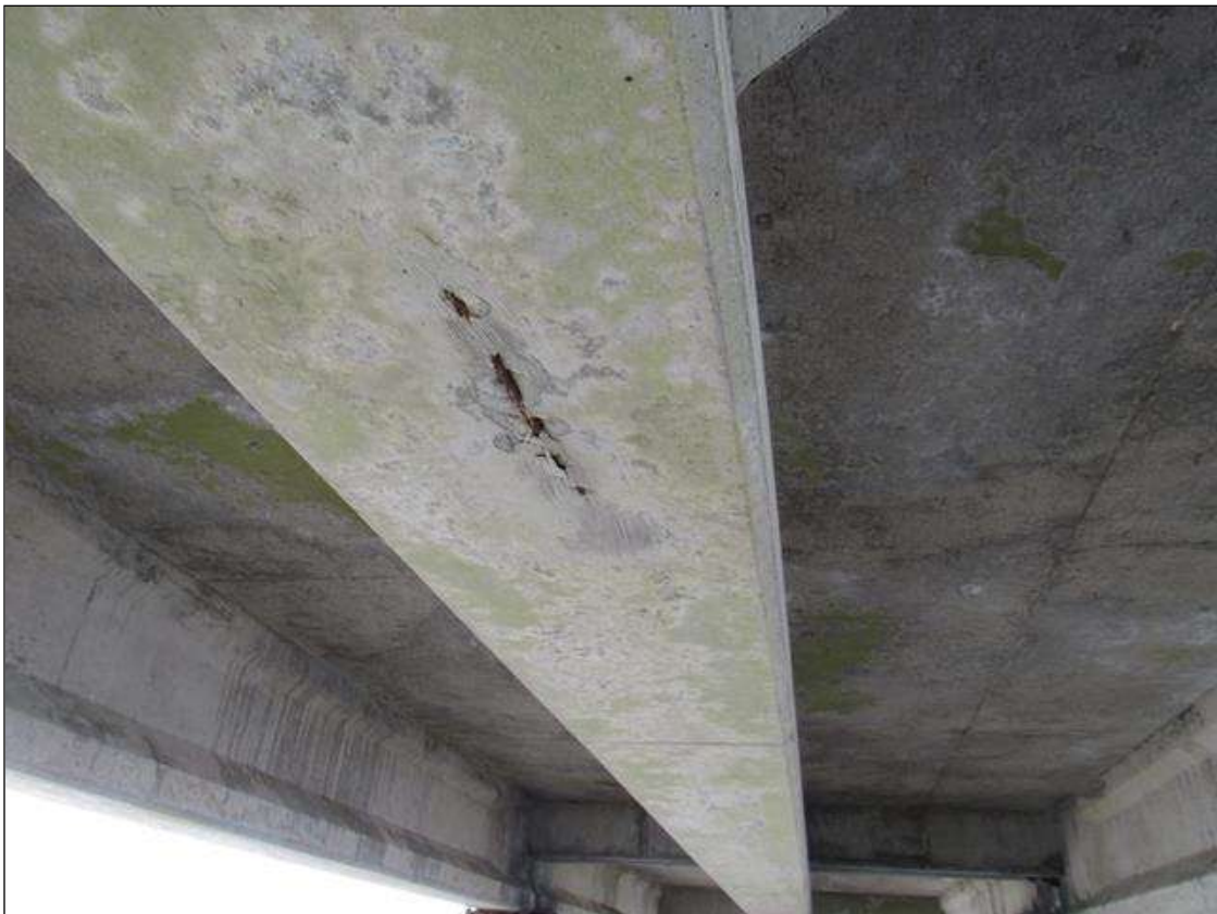
Span 65 Beam 3: 12" X 7" X UP TO 1/2" SPALL, WITH EXPOSED REINFORCING, BOTTOM FACE, NEAR MID SPAN.
