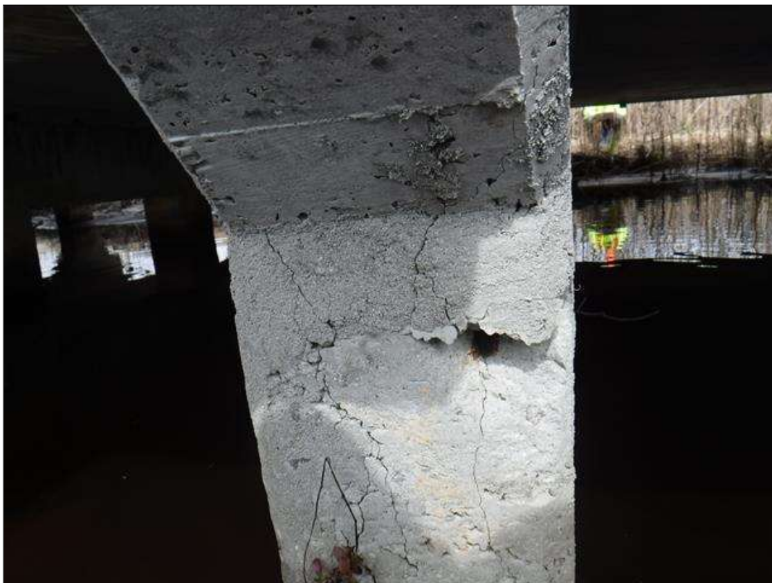
Bent 308 Pile 4: 5" X 8" X 4" FAILED PATCH AT BOTTOM SOUTH CORNER
