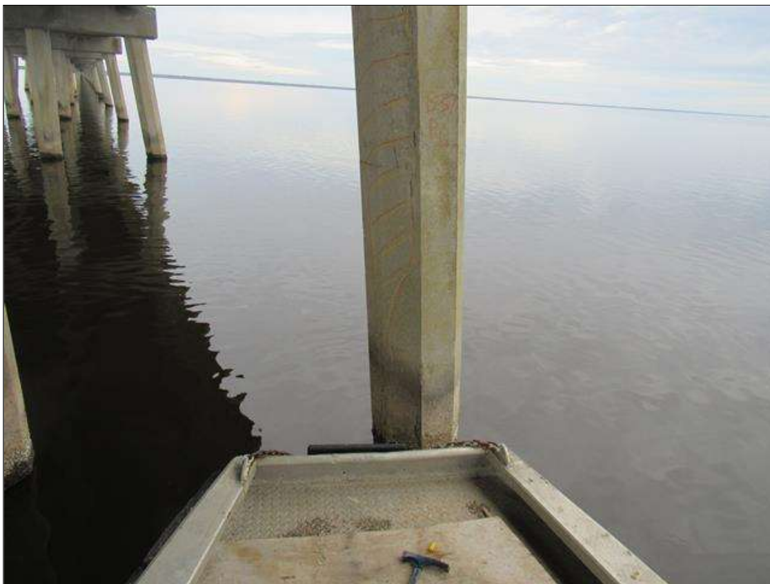
Bent 37 Saved Pile 6: 9.5' LONG X UP TO 22" WIDE DELAMINATION ON NORTH FACE, 3' FROM BOTTOM OF CAP.
