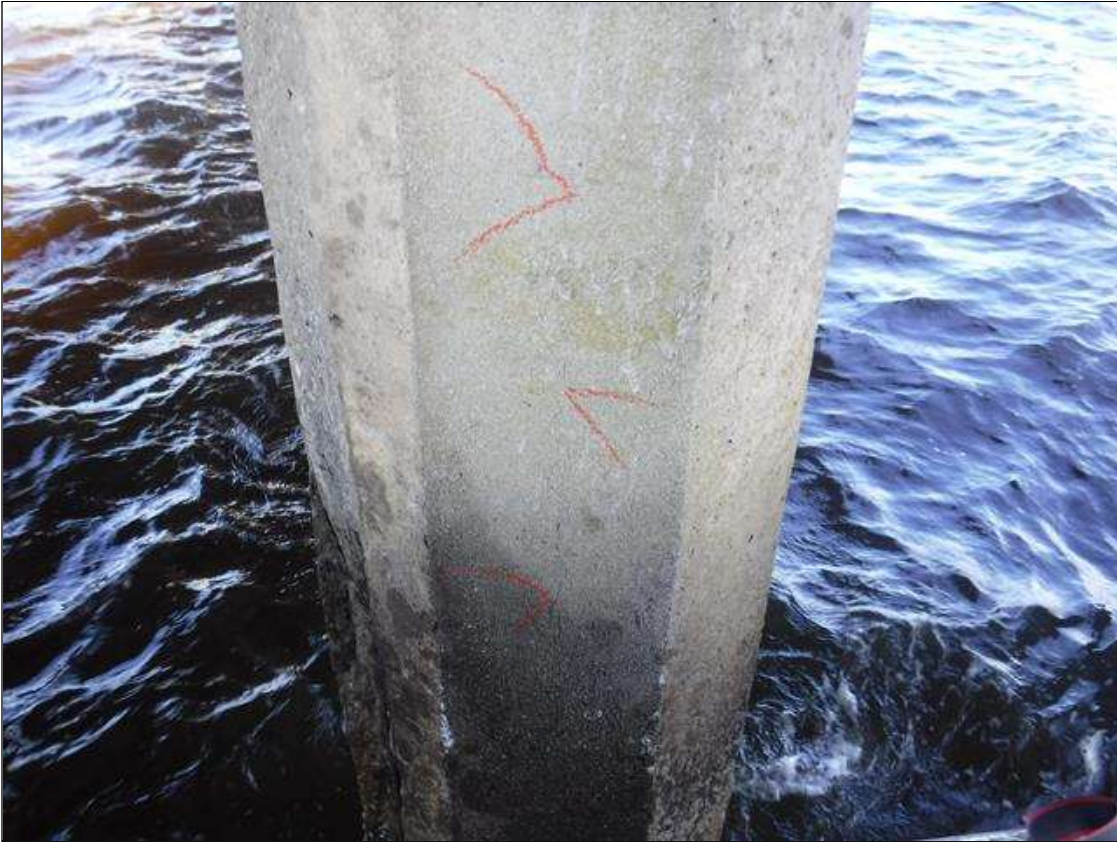
Bent 159 Pile 3: HAIRLINE CRACKS, 6' BELOW CAP, DOWN 10', MULTIPLE FACES. SCALING TO 1" DEEP WITH LOOSE AGGREGATE FROM WATERLINE TO MUDLINE.
