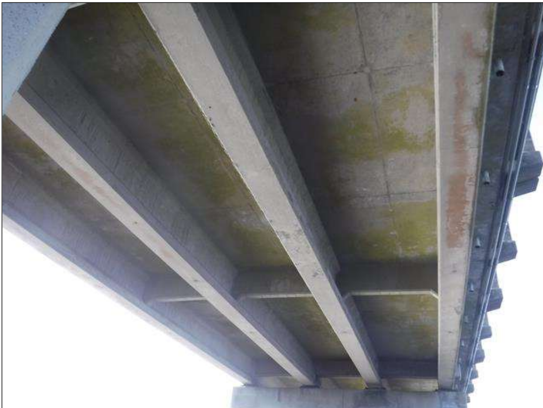
TYPICAL SUPERSTRUCTURE UNDERSIDE, SPAN 122 SHOWN
