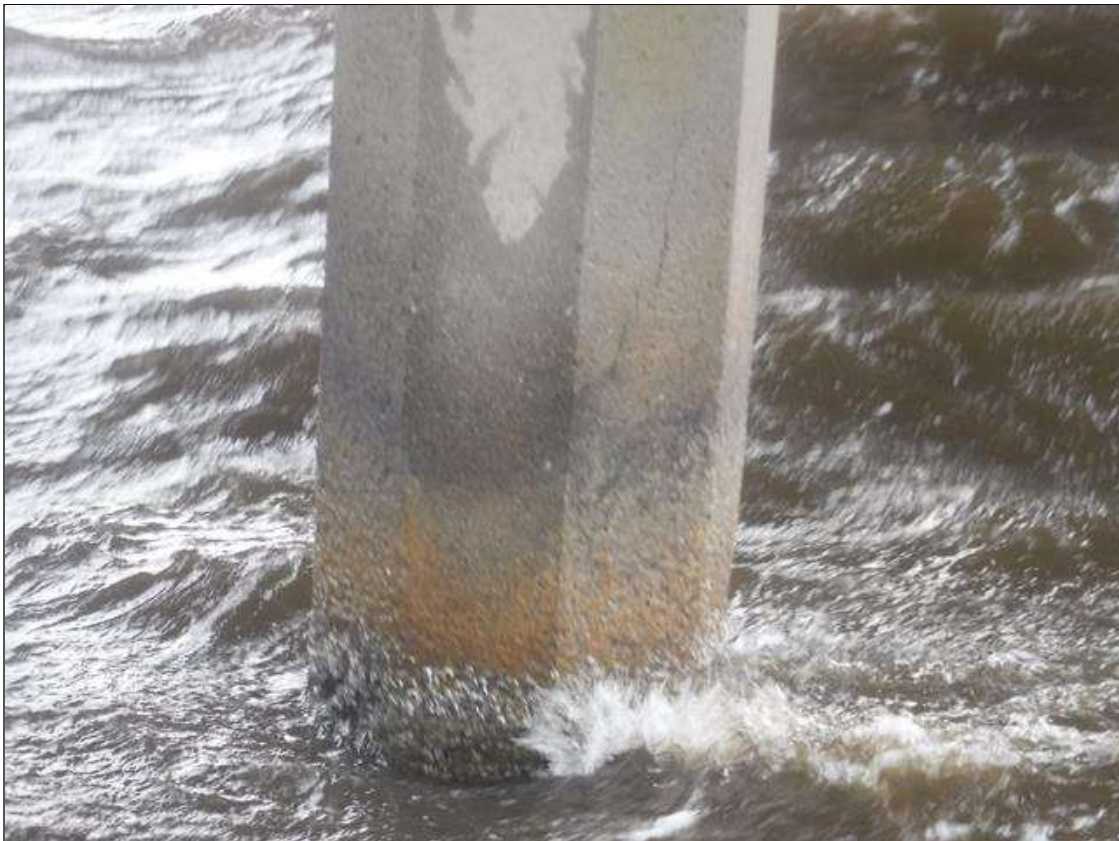
Bent 88 Pile 3: (PAR) (3) UP TO 3' X 0.06" VERTICAL CRACKS WITH 4' X 2' SURROUNDING DELAMINATION, ON WEST FACE, BEGINNING 8' BOTTOM OF CAP.
