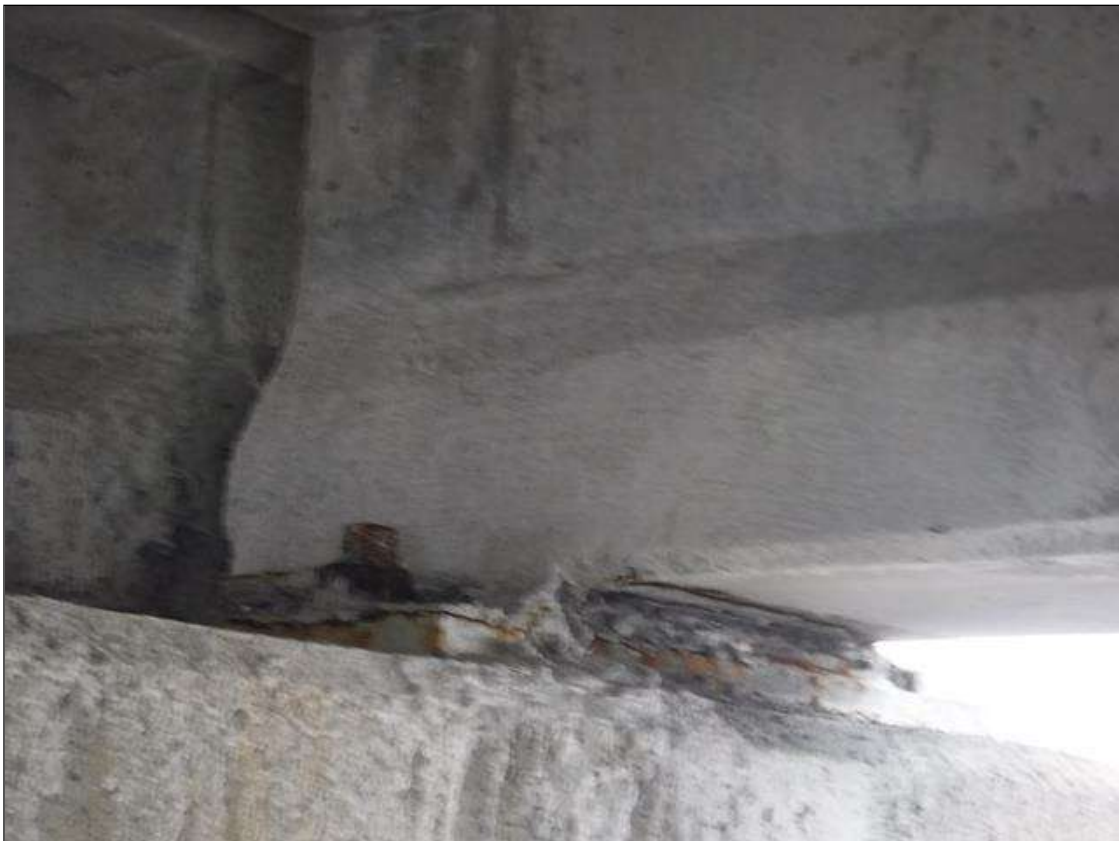
Span 199 Beam 4: 16" TALL X 16" LONG PATCHED AREA ON NORTH FACE AT BENT 199.
