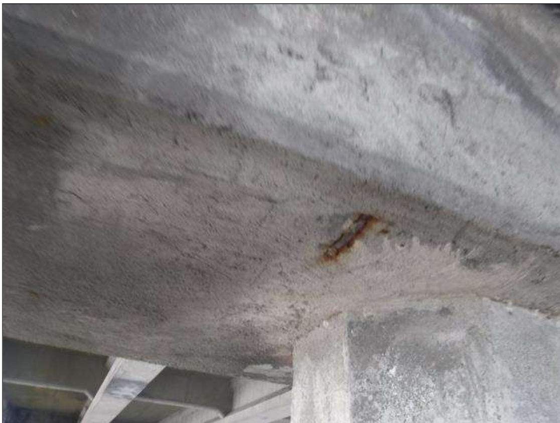
Bent 148 Cap 1: (2) 6" DIAMETER SPALLS WITH EXPOSED REBAR IN BOTTOM OF CAP BETWEEN PILES 3 AND
