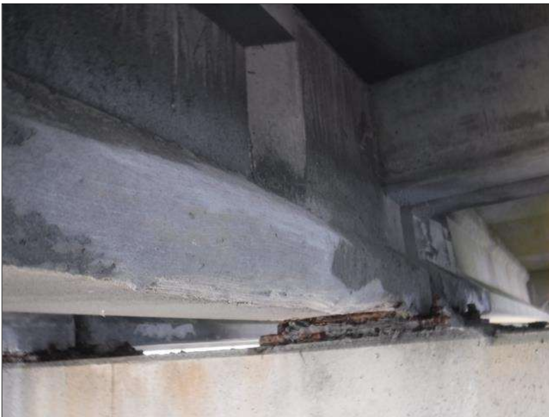
Span 21 Beam 2: 5' X 12" PATCH ON BOTTOM FLANGE, NORTH FACE, AT BENT 20.
