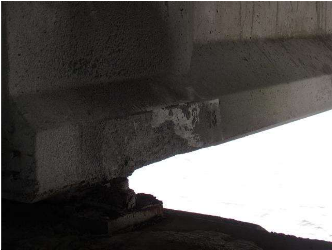
Span 38 Beam 2: 1' X 1' PATCHED AREA, SOUTH FACE, AT BENT 37.
