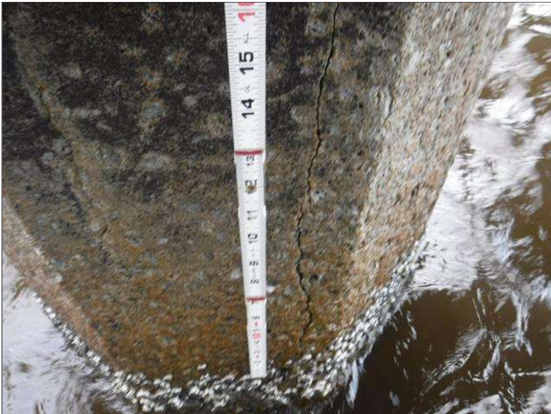
Bent 166 Pile 1: (PAR) HAIRLINE TO 1/16" CRACKS, 6' BELOW CAP, DOWN 10', MULTIPLE FACES. SCALING TO 1" DEEP WITH LOOSE AGGREGATE FROM WATERLINE TO MUDLINE.
