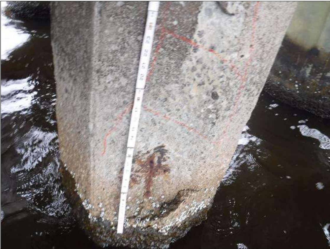
Bent 255 Pile 2: (PAR) 2' X UP TO 1' X 2.5" DEEP SPALL, WITH EXPOSED STRAND, SOUTH FACE, 8' FROM BOTTOM OF CAP.
