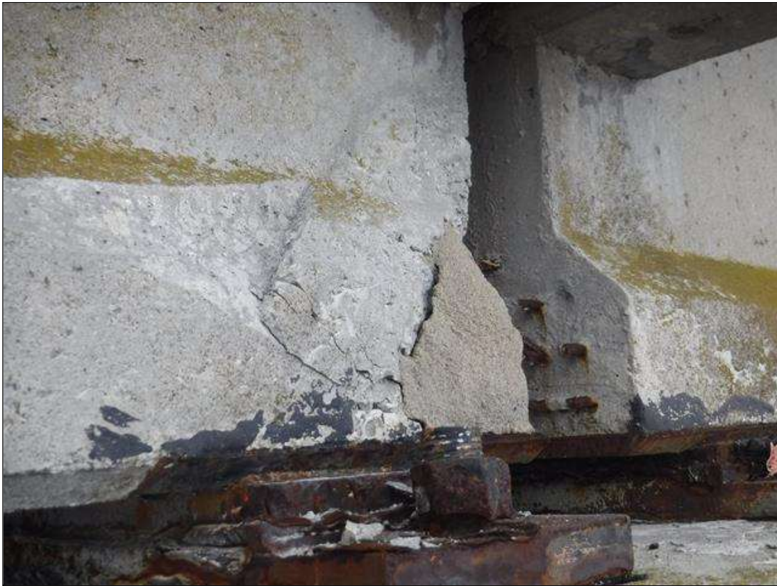
Span 182 Beam 1: (PAR) 18" X 10" X 5" SPALL, WITH EXPOSED PRESTRESSING, NORTH FACE, AT BENT 181.
