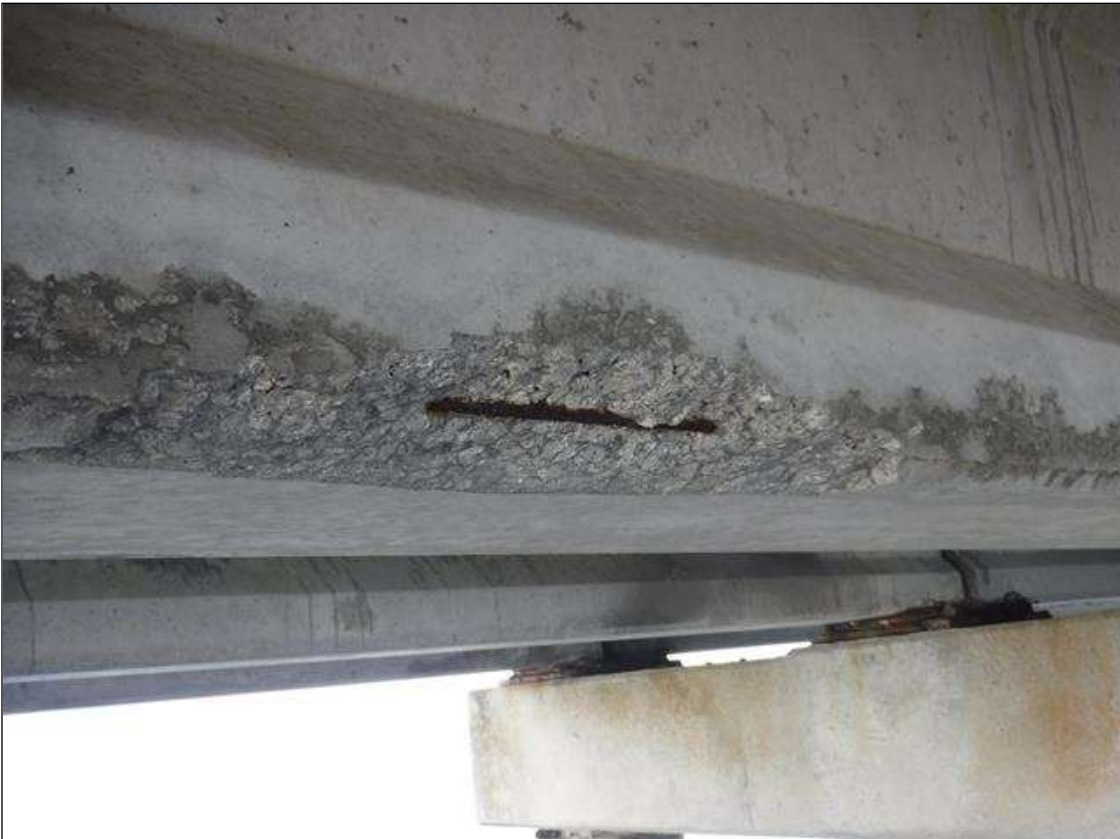
Span 121 Beam 2: (PAR) 30" X 3" X 3" EDGE SPALL, WITH EXPOSED STRAND, BOTTOM NORTH CORNER, 12' FROM BENT 120.
