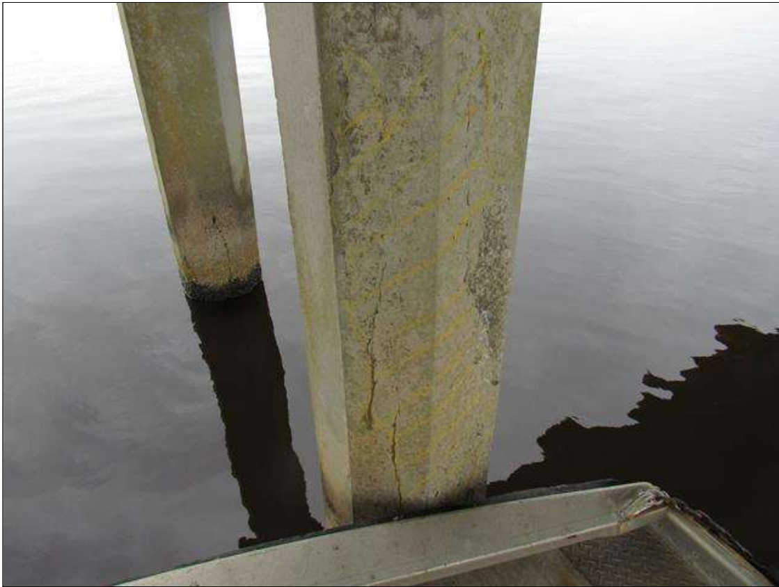
Bent 34 Saved Pile 2: (PAR) HAIRLINE TO 1/8" CRACK WITH 7' X 16" ADJACENT DELAMINATION, 6' BELOW CAP, DOWN 8', SOUTH FACS. SCALING TO 1" DEEP WITH LOOSE AGGREGATE FROM WATERLINE TO MUDLINE.
