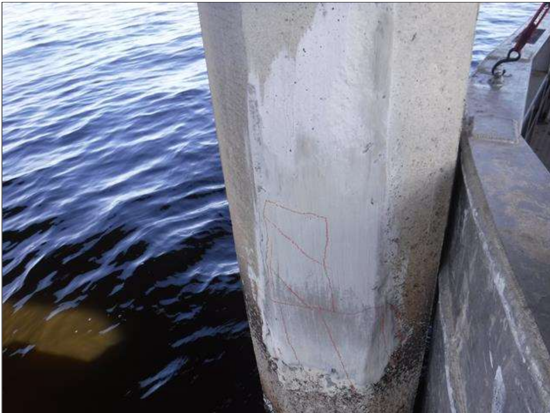
Bent 218 Pile 3: 4' X 2' FAILED PATCHED AREA ON SOUTH FACE WITH BOTTOM 12" DELAMINATED, 7' FROM BOTTOM OF CAP.
