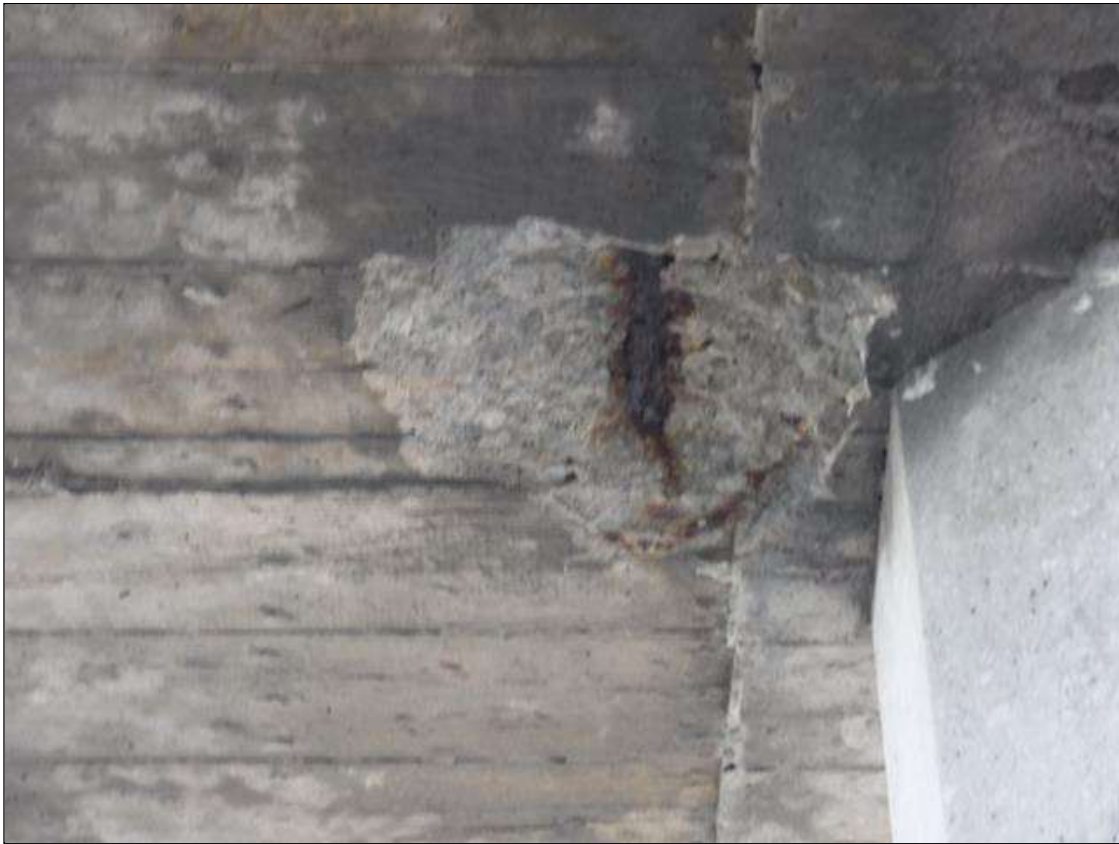
Bent 166 Cap 1: (PAR) 1' X 1' X 1" SPALL, WITH EXPOSED PRIMARY REINFORCEMENT, BOTTOM OF CAP, NORTH OF PILE 2. REBAR HAS 10% SECTION LOSS
