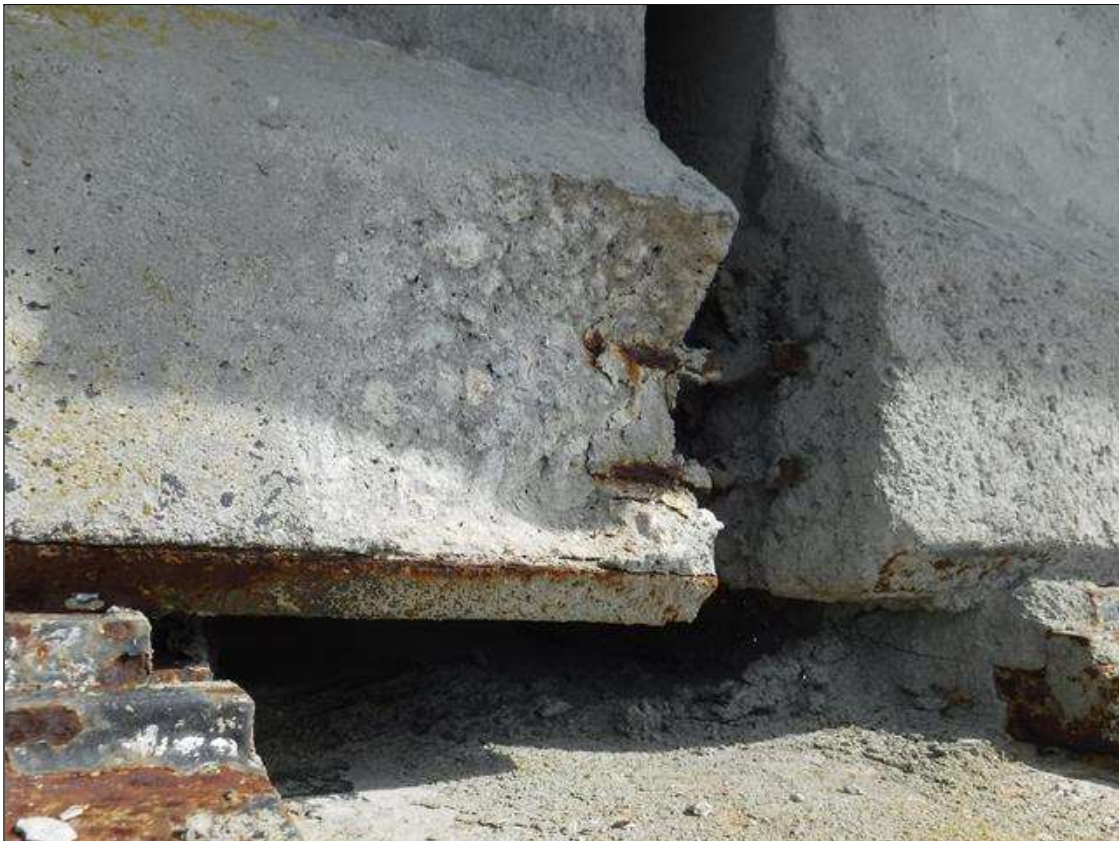
Span 224 Beam 4: (PAR) 6" X 6" X 3" DEEP SPALL WITH EXPOSED STRAND ON BOTTOM FLANGE SOUTH FACE AT BENT 224
