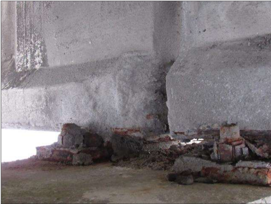
Span 56 Beam 4: 12" X 12" PATCHED AREA, NORTH FACE, AT BENT 55.
