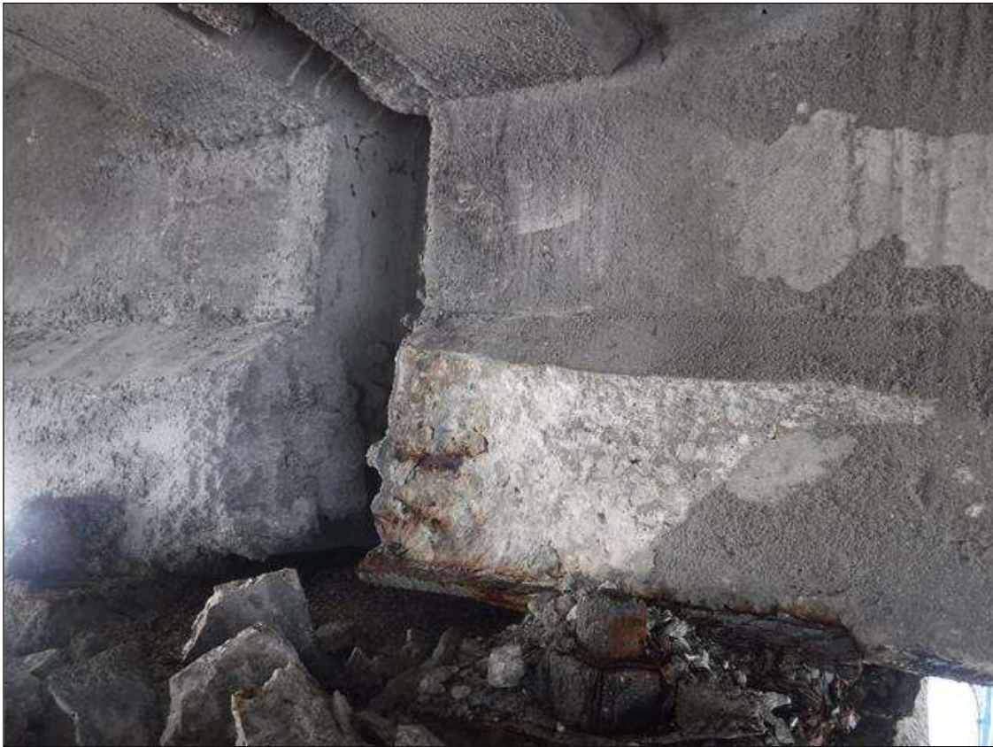
Span 76 Beam 3: (PAR) 15" X 6" X 3" DEEP SPALL WITH EXPOSED STRAND ON SOUTH FACE AT BENT 76
