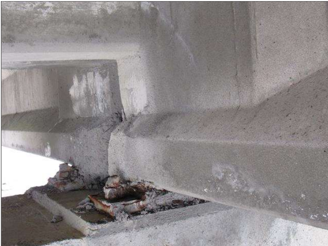
Span 37 Beam 3: 4' X UP TO 18" PATCHED AREA, BOTTOM FACE, EXTENDING 10" ONTO NORTH AND SOUTH FACES, AT BENT 36.
