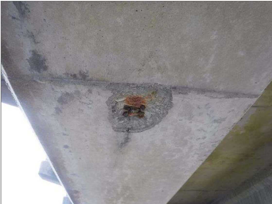
Span 216 Beam 1: 6" DIAMETER X 1/2" DEEP SPALL WITH EXPOSED REBAR ON BOTTOM FACE AT MIDSPAN
