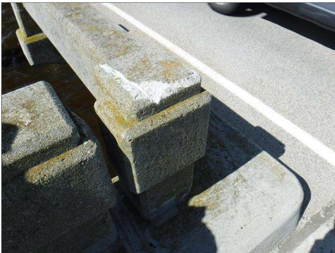
Span 114 Right Bridge Rail: 10" X 5" X 1 1/2" ABRASION AT TOP RIGHT CORNER OF POST 9
