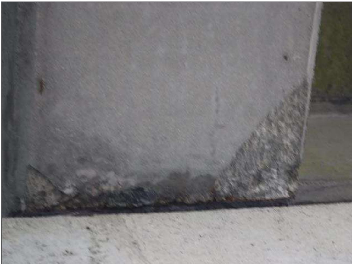
Span 174 Beam 3: 6" X 6" X 1" SPALL, BOTTOM OF BEAM, AT BENT 174.
