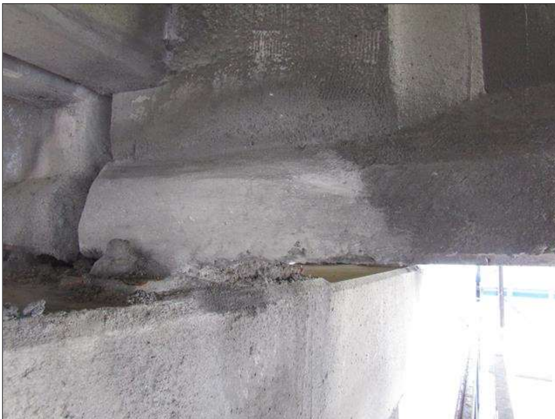
Span 36 Beam 3: 2' X 1" PATCHED AREA, BOTTOM FACE, EXTENDING 1' ONTO SOUTH FACE, AT BENT 36.
