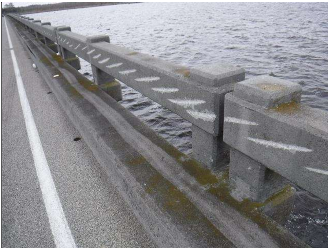
Span 258 Right Bridge Rail: 42' OF SCRAPES AND GAUGES CAUSED BY IMPACT DAMAGE ON LEFT FACE LOCATED ALONG RAIL
