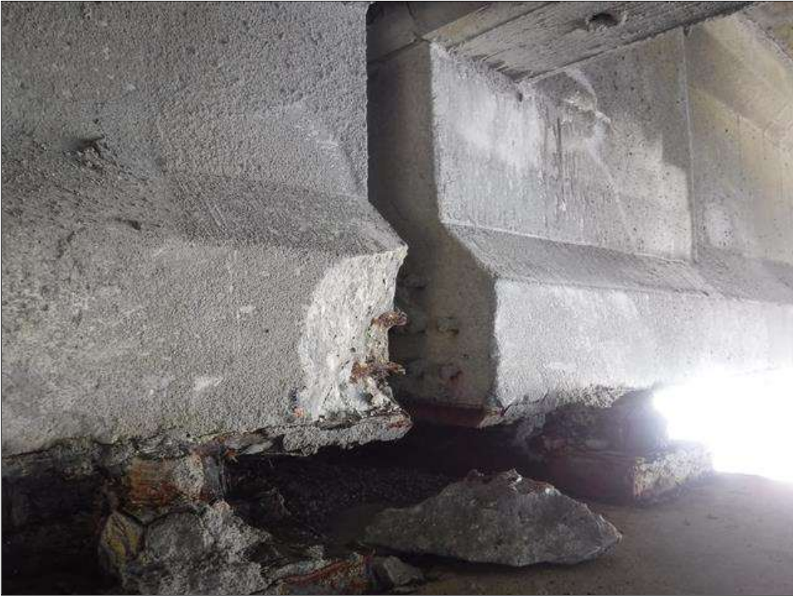
Span 118 Beam 2: (PAR) 6" X 6" X 2" DEEP SPALL WITH EXPOSED STRAND ON SOUTH FACE AT BENT 118
