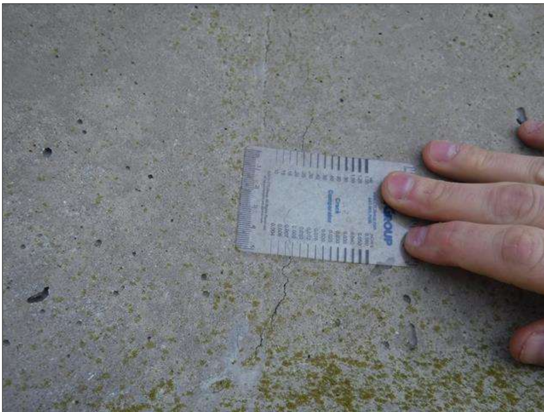
Span 139 Beam 4: 16" X 0.009" VERTICAL CRACK, EAST FACE, 3' FROM BENT 138.
