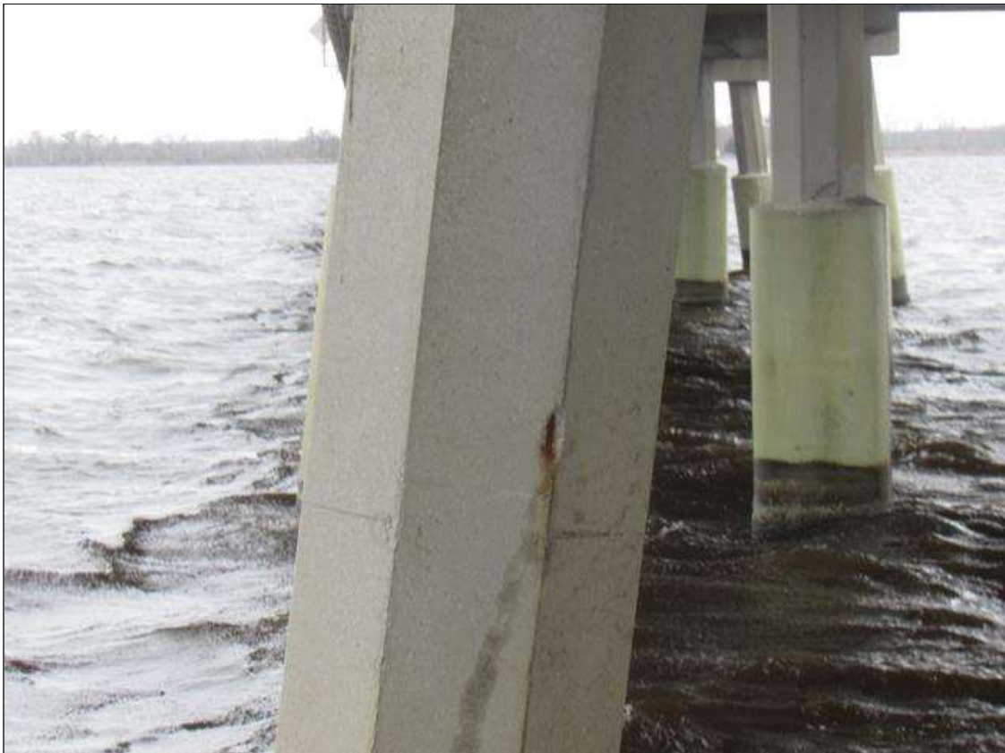
Bent 107 Pile 4: 4" X 2" X 1 1/2" SPALL, WITH EXPOSED REINFORCING, EAST FACE, 6' FROM BOTTOM OF CAP.
