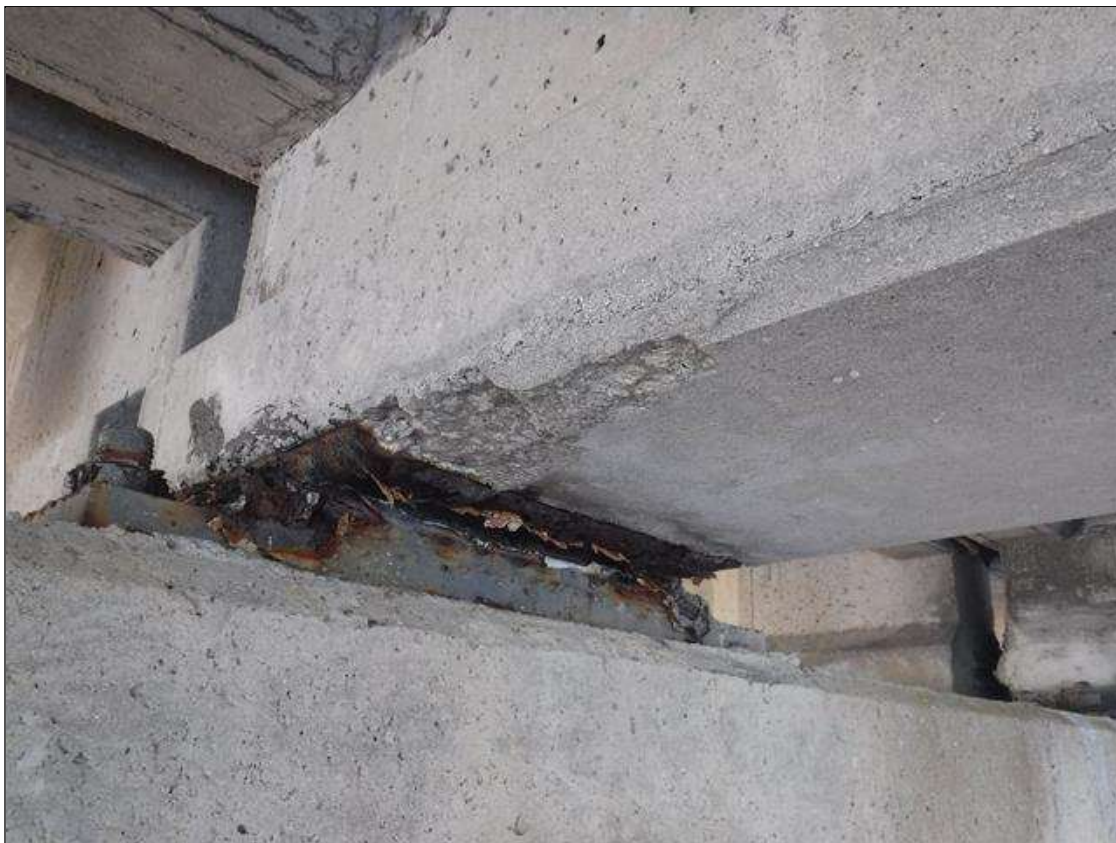
Span 121 Beam 2: 10" X 3" X 1/2" DEEP SPALL ON BOTTOM NORTH FACE AT BENT 121
