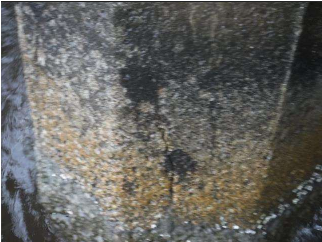
Bent 86 Pile 1: (PAR) (2) UP TO 3' X 0.03" VERTICAL CRACKS, BEGINNING 8' BOTTOM OF CAP, AT RANDOM THROUGHOUT.
