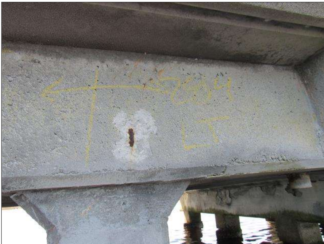
Span 284 Deck: 4" DIAMETER X 1/2" DEEP SPALL WITH EXPOSED REBAR ON LEFT FACE LOCATED ABOVE BENT 284
