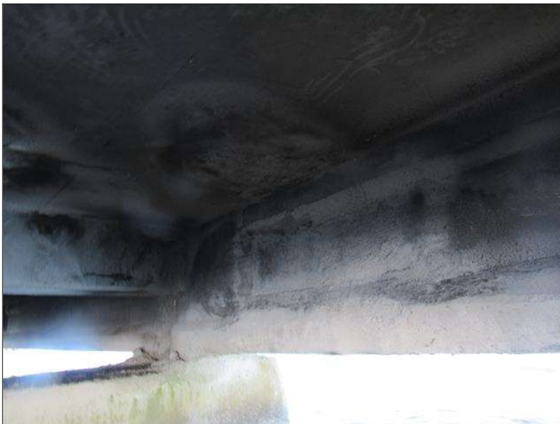
Span 3 Beam 1: 12' X UP TO 32" PATCHED AREAS, AT RANDOM THROUGHOUT, NORTH AND SOUTH FACES, BEGINNING AT BENT 2.
