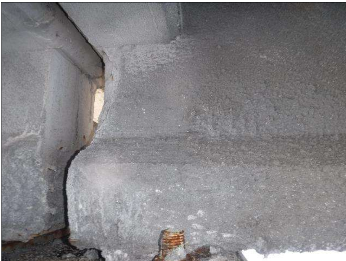
Span 11 Beam 2: 12" TALL, 6" LONG PATCHED AREA ON BOTH SIDES OF GIRDER AT BENT 11.
