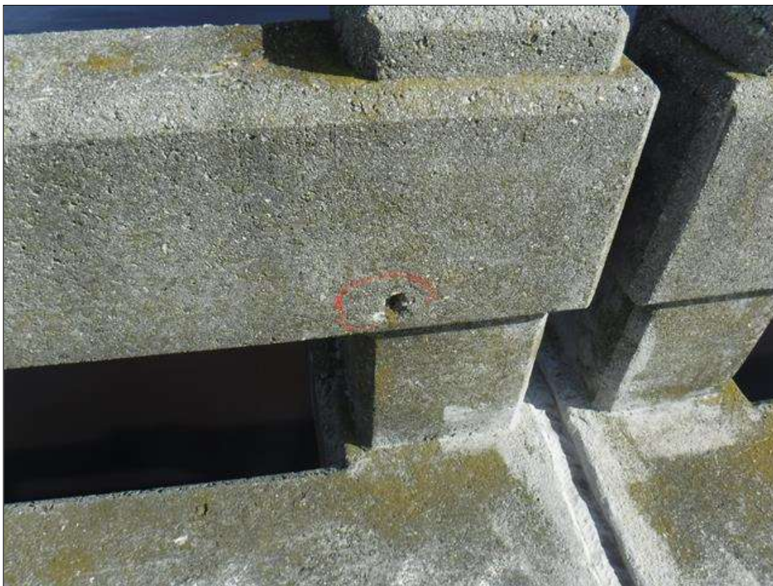
Span 268 Left Bridge Rail: 2" DIAMETER X 1/2" DEEP SPALL WITH EXPOSED REBAR ON RIGHT FACE ON POST 9
