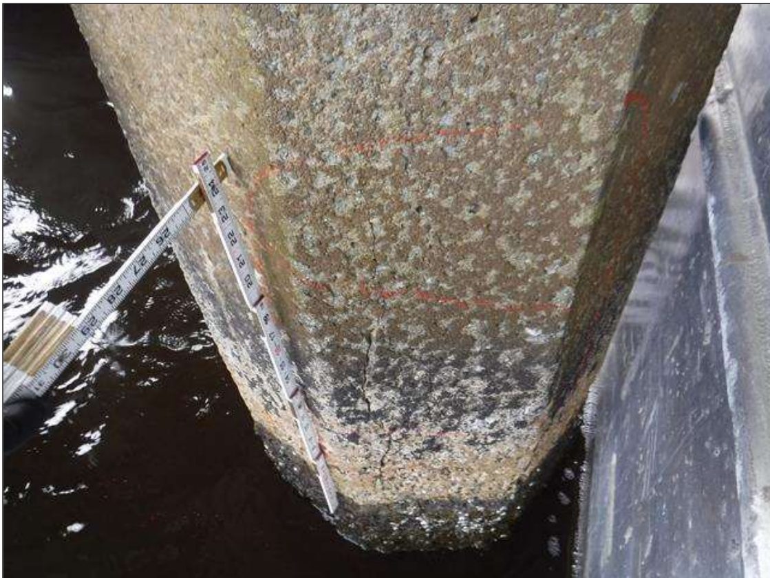
Bent 227 Pile 2: (PAR) (3) UP TO 2' X 0.04" VERTICAL CRACKS, NORTH FACE, 8' FROM BOTTOM OF CAP, WITH ADJACENT 2' X 2' DELAMINATION.
