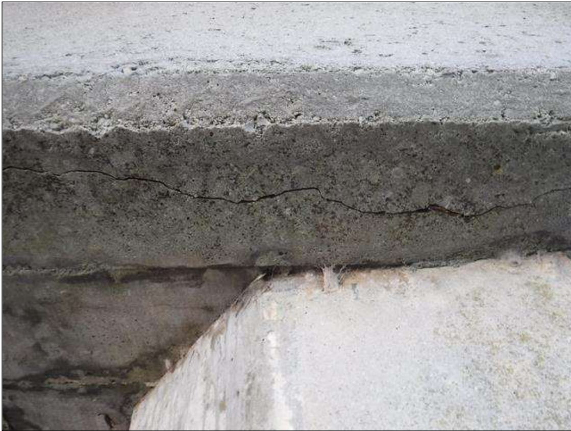
Bent 160 Cap 1: 10' LONG X 1/16" LONGITUDINAL CRACK ON BOTTOM EAST FACE OF CAP AT PILE 1
