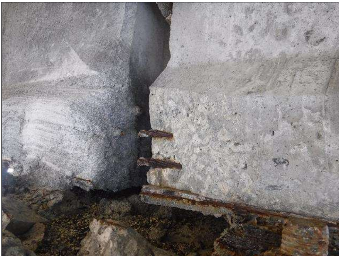
Span 140 Beam 3: (PAR) 8" X 8" X 3" SPALL, WITH EXPOSED STRAND, NORTH FACE, AT BENT 140.
