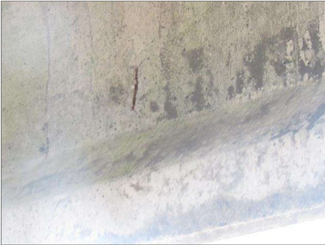
Span 6 Beam 4: 1" X 6" X 1/2" SPALL, WITH EXPOSED REINFORCING, NORTH FACE, 3' FROM BENT 6.
