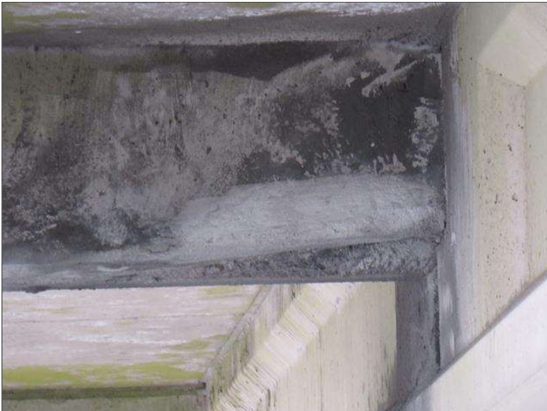
Span 52 Beam 1: 18" X 12" X 12" CORNER PATCHED AREA, END DIAPHRAGM, BETWEEN BEAMS 1 AND 2, EAST
