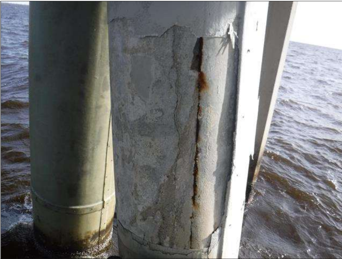
Bent 127 Pile 4: PILE HAS BEEN JACKETED, BEGINNING 1' FROM BOTTOM OF CAP, WITH PILE JACKET MISSING, AT RANDOM THROUGHOUT, EXTENDING BELOW WATERLINE, WITH EXPOSED REINFORCING.
