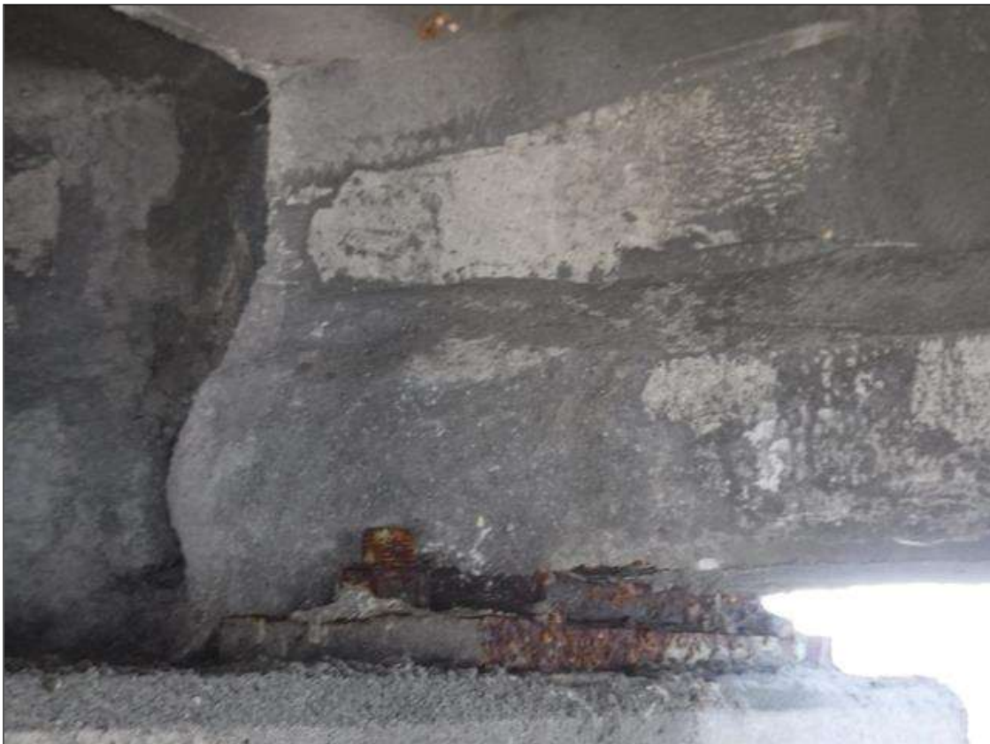
Span 21 Beam 1: (2) UP TO 24" X 12" PATCHED AREAS, NORTH AND SOUTH FACES, AT BENT 20.
