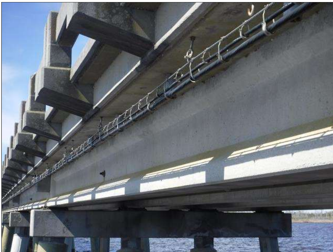
UTILITY ALONG SOUTH OVERHANG, SPAN 6 SHOWN
