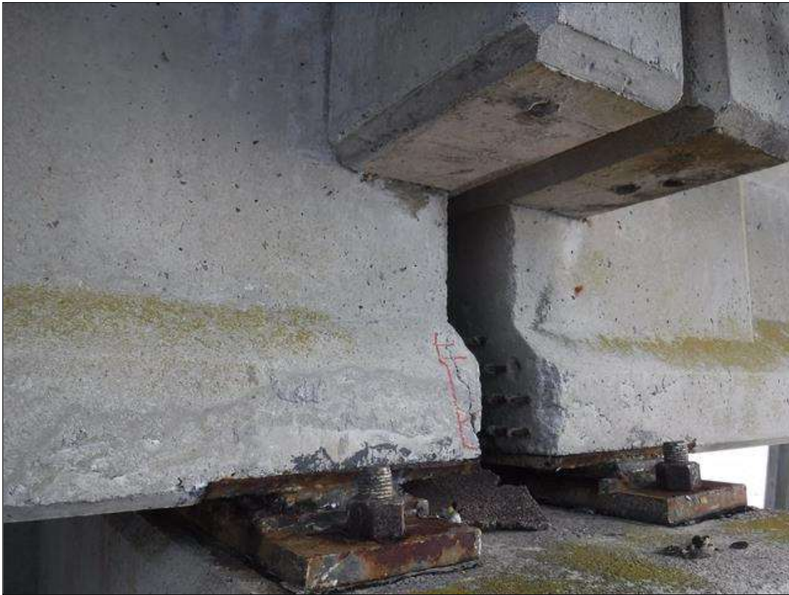
Span 73 Beam 4: 18" X 9" DELAMINATION, SOUTH FACE, AT BENT 73.
