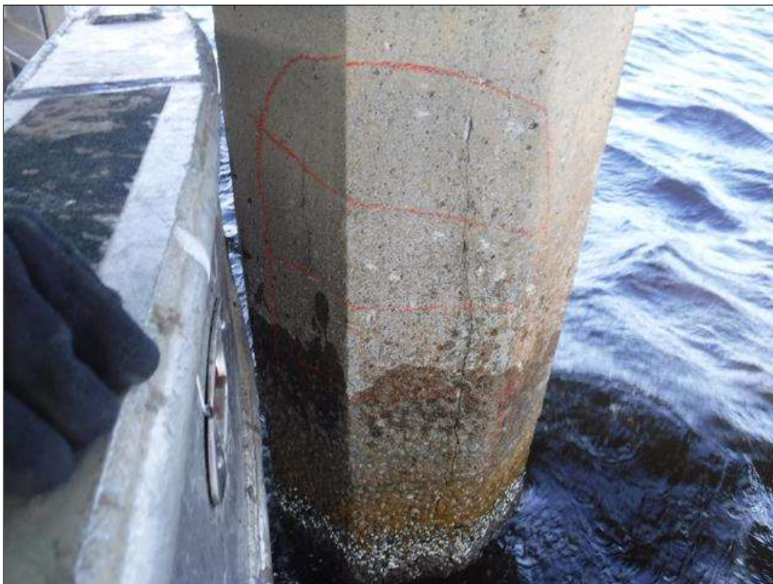
Bent 128 Pile 2: 3' X 2' DELAMINATION, SOUTH FACE, 8' FROM BOTTOM OF CAP, EXTENDING BELOW WATERLINE.
