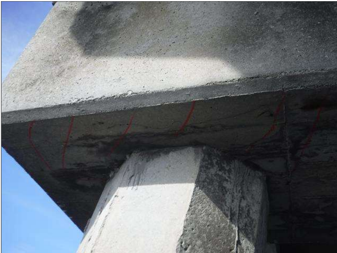
Bent 157 Cap 1: 4' X 18" DELAMINATION ON BOTTOM OF CAP AT PILE 4
