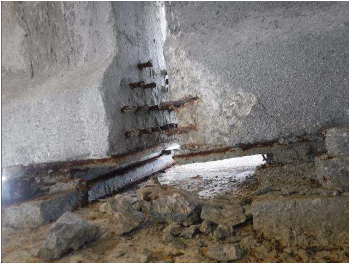
Span 205 Beam 4: (PAR) 6" X 6" X 2" DEEP SPALL WITH EXPOSED STRANDS IN BOTTOM FLANGE, NORTH FACE AT BENT 205
