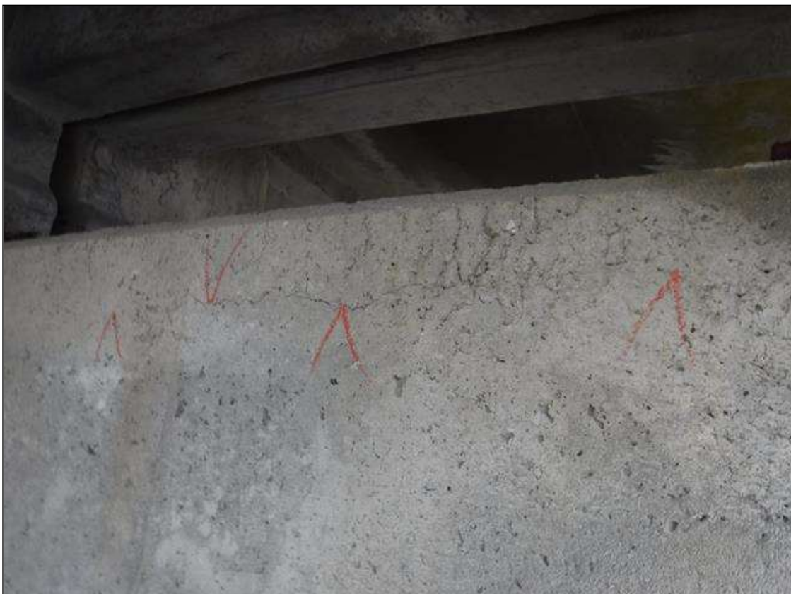
Bent 189 Cap 1: 3' HAIRLINE CRACK ON EAST FACE BETWEEN BEAM 1 AND 2
