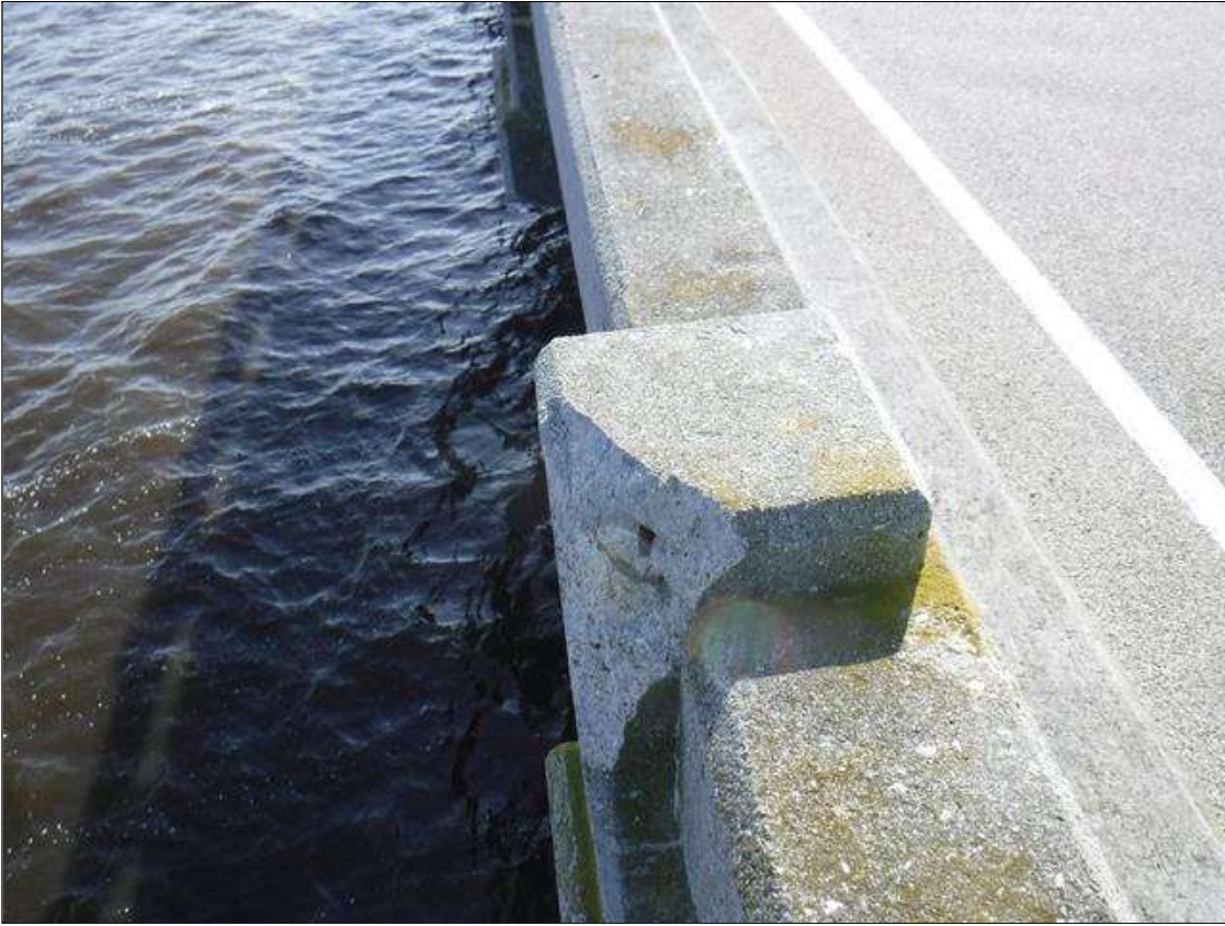
Span 143 Left Bridge Rail: 8" X 6" X 12" SPALL WITH EXPOSED REBAR AT TOP LEFT CORNER LOCATED ON POST 2
