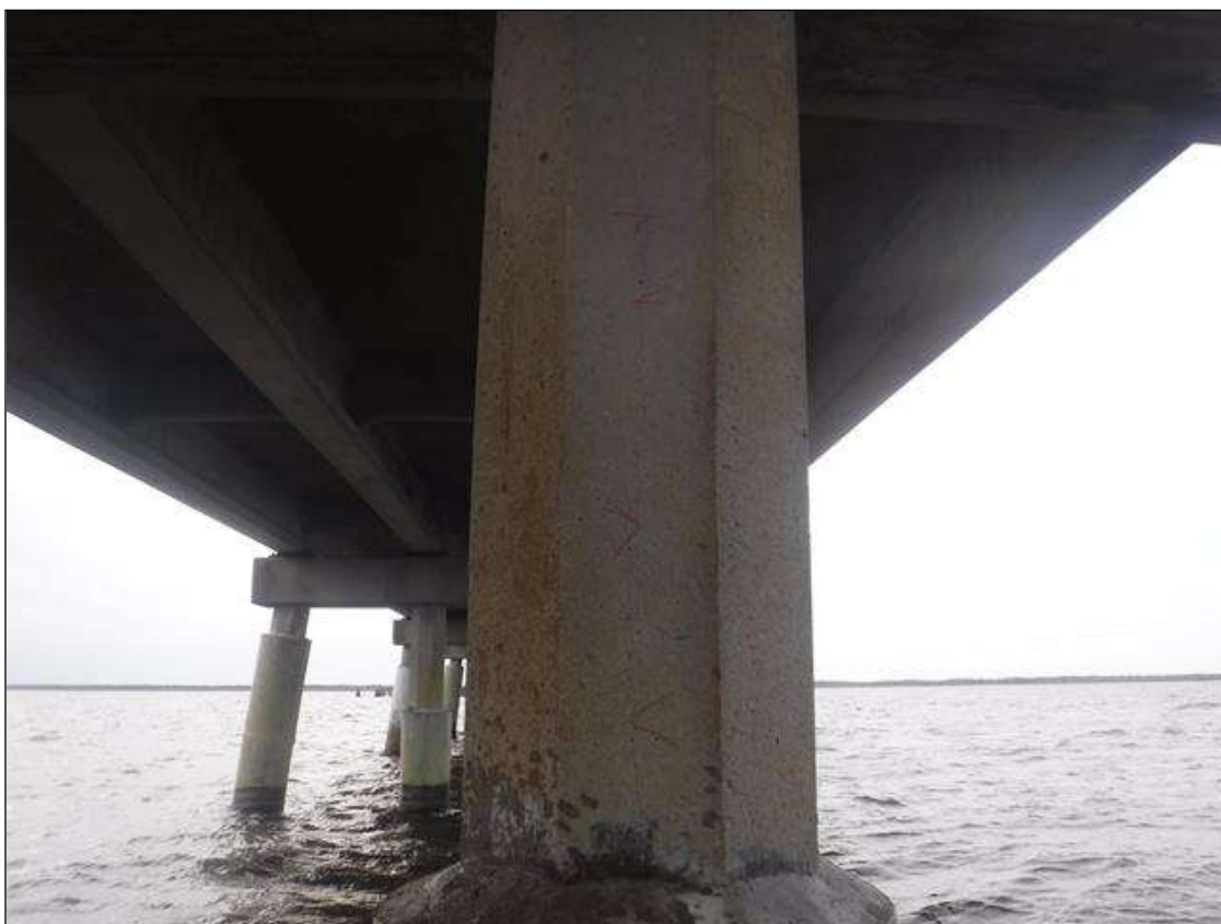
Bent 138 Pile 2: (PAR) UP TO 5' X 0.013" VERTICAL CRACKS ON EAST FACE, BEGINNING AT BOTTOM OF CAP.
