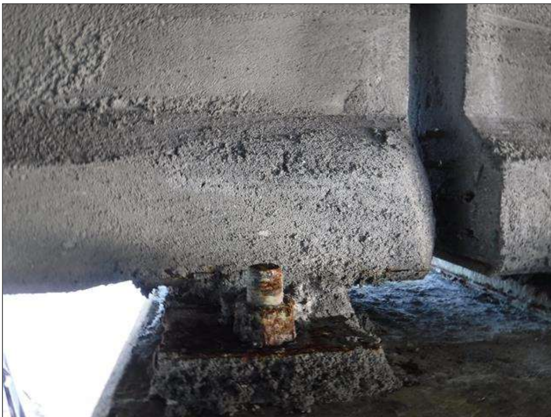
Span 10 Beam 1: PATCHED AREA IN GIRDER IN BOTTOM BULB OVER BENT 10 BEARING SOUTH FACE.
