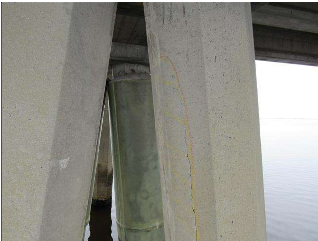
Bent 37 Saved Pile 5: 9' X UP TO 4' WIDE DELAMINATION ON WEST, SOUTH AND EAST FACES LOCATED AT 18' FROM BOTTOM OF CAP
