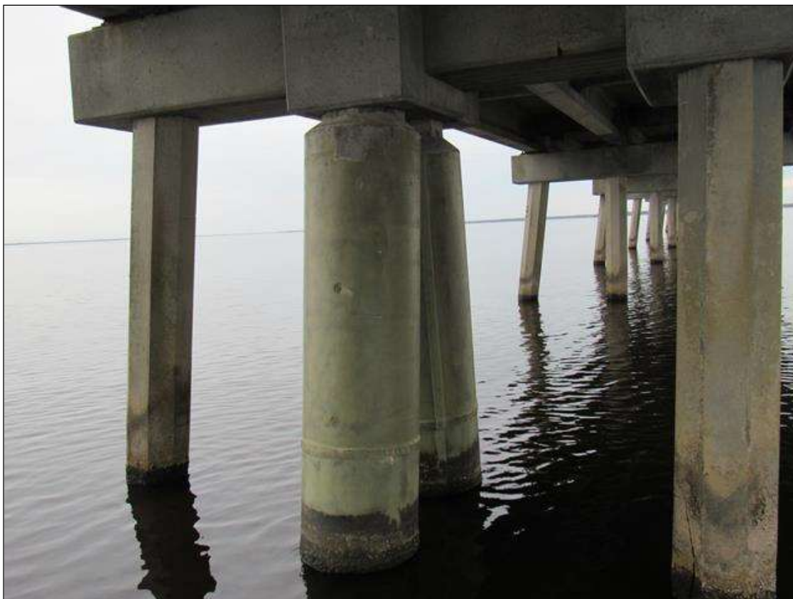
Bent 37 Saved Pile 2: PILE HAS BEEN JACKETED, BEGINNING 1' FROM BOTTOM OF CAP AND EXTENDING BELOW WATERLINE.
