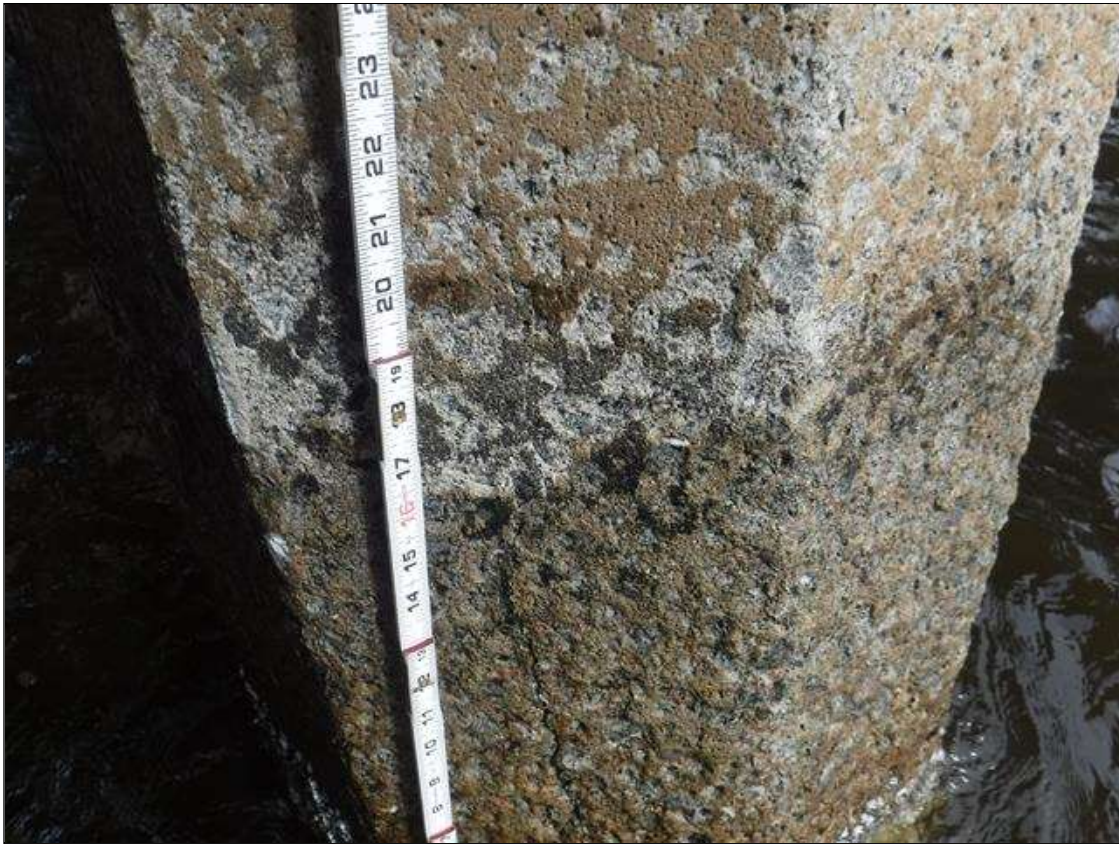
Bent 179 Pile 6: (PAR) HAIRLINE TO 1/4" CRACKS, 8' BELOW CAP, DOWN 4' , MULTIPLE FACES. SCALING TO 1" DEEP WITH LOOSE AGGREGATE FROM WATERLINE TO MUDLINE.
