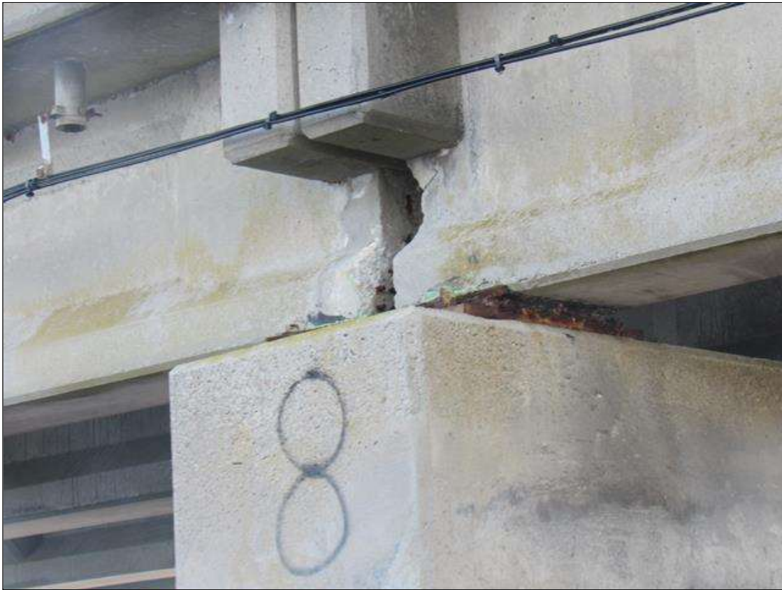
Span 9 Beam 1: (PAR) 12" X 6" X UP TO 3" DEEP SPALL WITH EXPOSED STRAND, WEST FACE, AT BENT 8.
