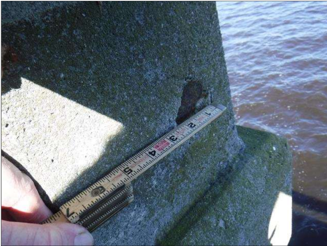
Span 31 Left Bridge Rail: 3" DIAMETER SPALL ON NEAR FACE LOCATED 5TH POST FROM BENT 30
