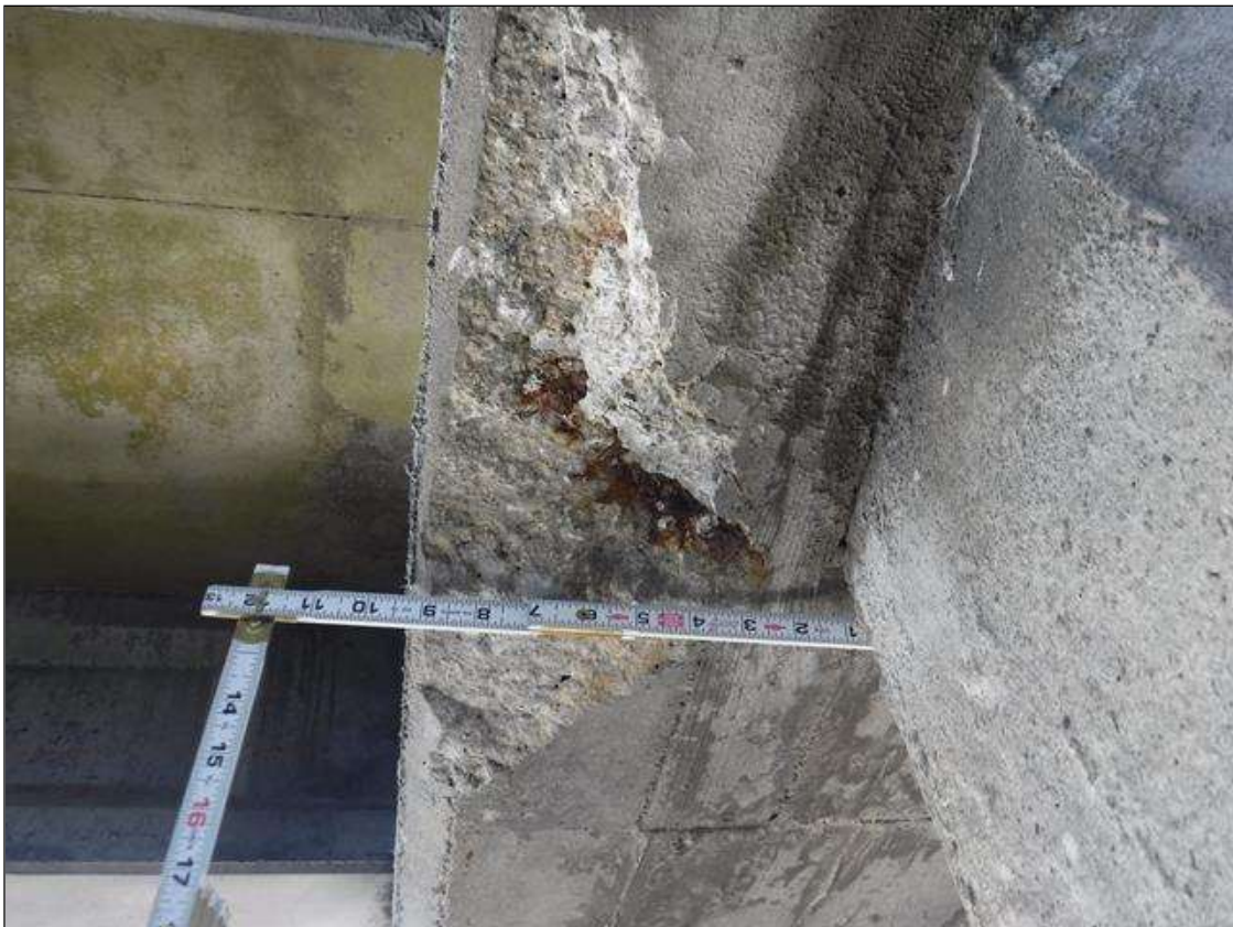
Bent 218 Cap 1: (PAR) 18" X UP TO 7" X 1.5" SPALL, WITH EXPOSED PRIMARY REINFORCING, BOTTOM OF CAP, AT PILE 3. REBAR HAS MINOR SECTION LOSS.
