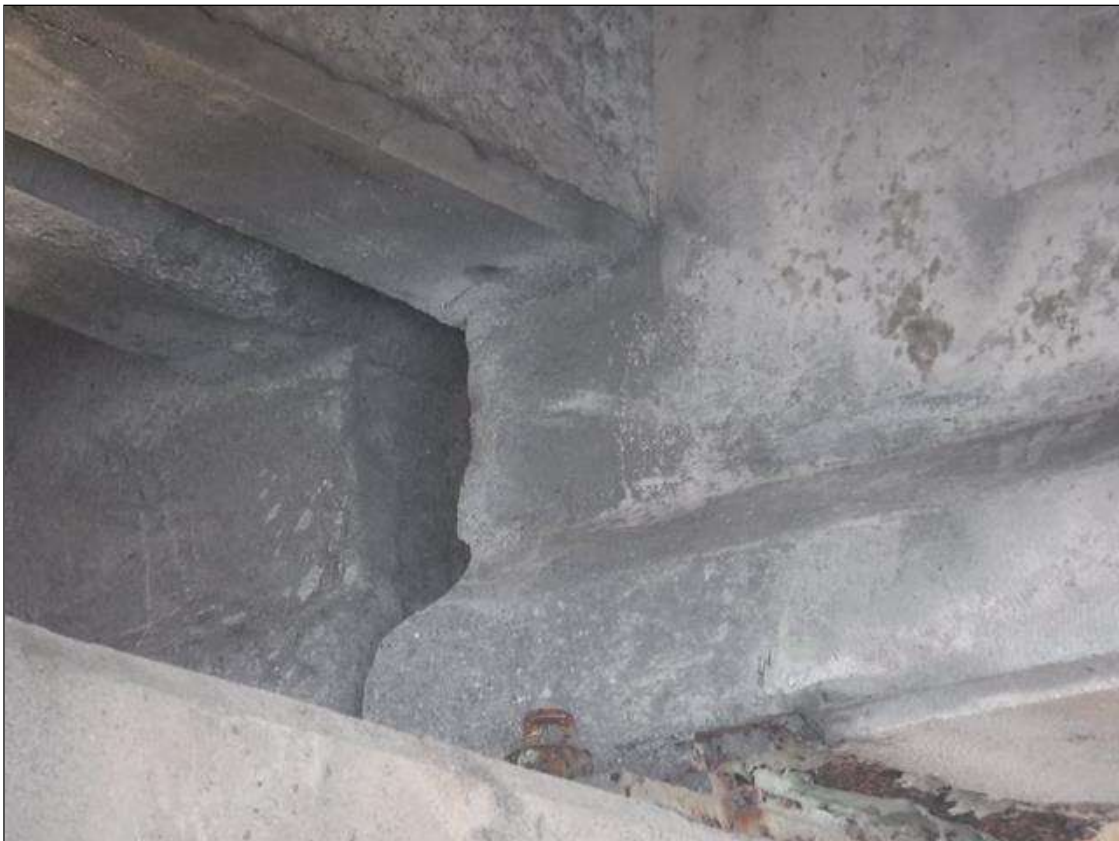
Span 15 Beam 3: (2) UP TO 12" X 18" PATCHED AREAS, NORTH AND SOUTH FACES, AT BENT 15.
