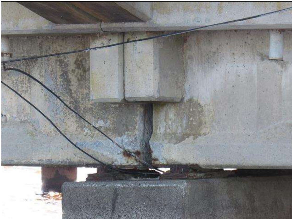
Span 2 Beam 1: (PAR) 18" X 8" X 2" SPALL, WITH EXPOSED STRAND, NORTH FACE, AT BENT 1.
