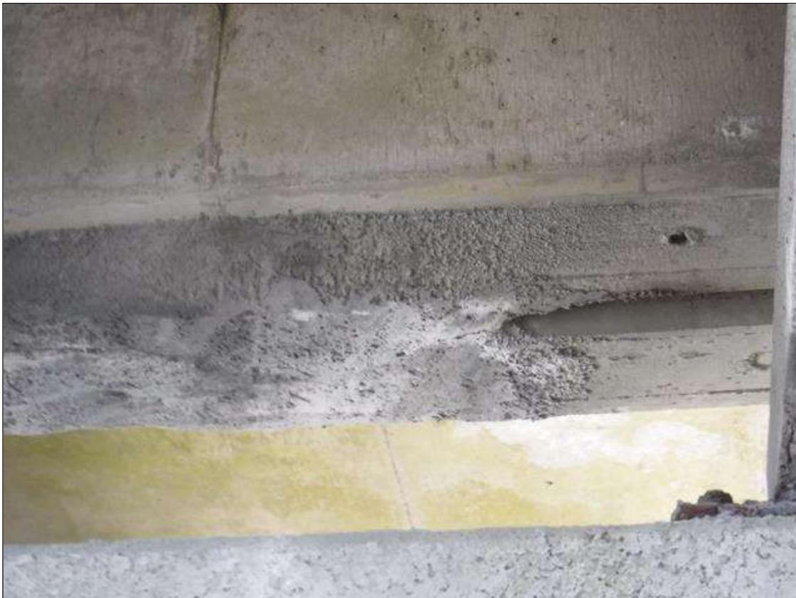
Span 118 Beam 3: 5' X UP TO 1' PATCHED AREA, WEST FACE OF BENT 118 DIAPHRAGM, BETWEEN BEAMS 2 AND 3.
