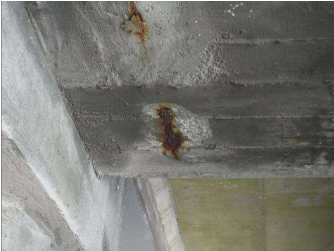
Bent 127 Cap 1: 12" X 1" DEEP SPALL WITH EXPOSED REBAR ON BOTTOM FACE, RIGHT OF PILE 2
