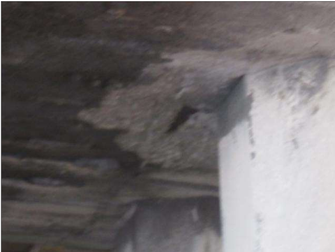
Bent 115 CAP REST PIER 1: 2' X 2' X 1" DEEP SPALL WITH EXPOSED REBAR BOTTOM FACE NEAR PILE 11.
