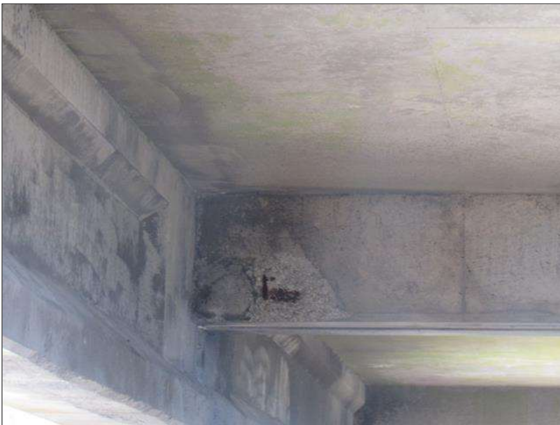
Span 5 Beam 4: 2' X 1' SPALLED PATCHED AREA, WITH EXPOSED REINFORCING, EAST FACE OF BENT 4 DIAPHRAGM, BETWEEN BEAMS 3 AND 4.
