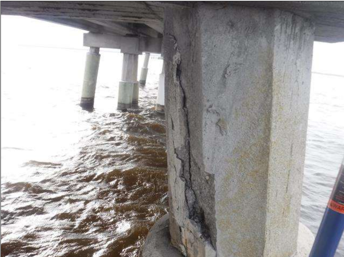
Bent 136 Saved Pile 1: (PAR) 36" X 20" DELAMINATION AND 3" DEEP SPALL WITH 2" OF EXPOSED STRAND, SOUTH FACE, BEGINNING AT BOTTOM OF CAP.
