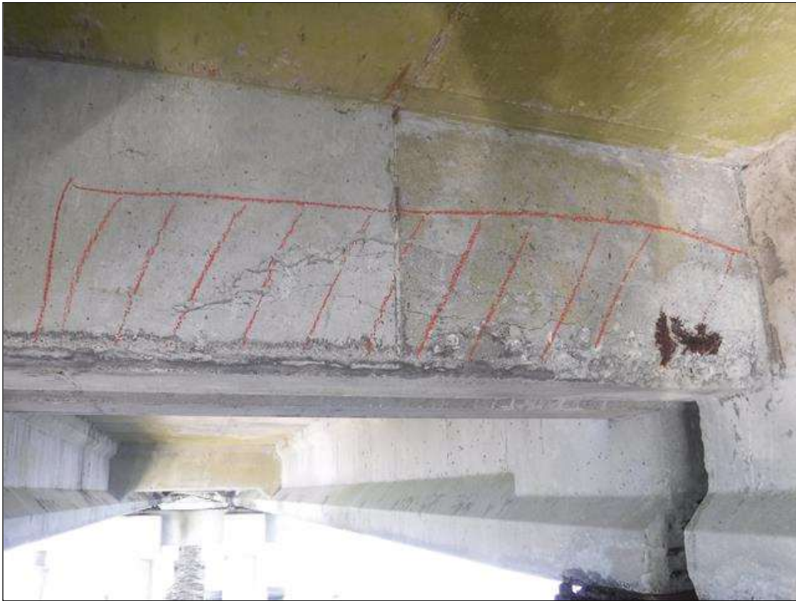
Span 137 Beam 2: (PAR) 18" X UP TO 12" X 1" SPALL, WITH EXPOSED REINFORCING, EAST FACE, BENT 136 DIAPHRAGM, BETWEEN BEAMS 2 AND 3, WITH 4' X 12" DELAMINATION.
