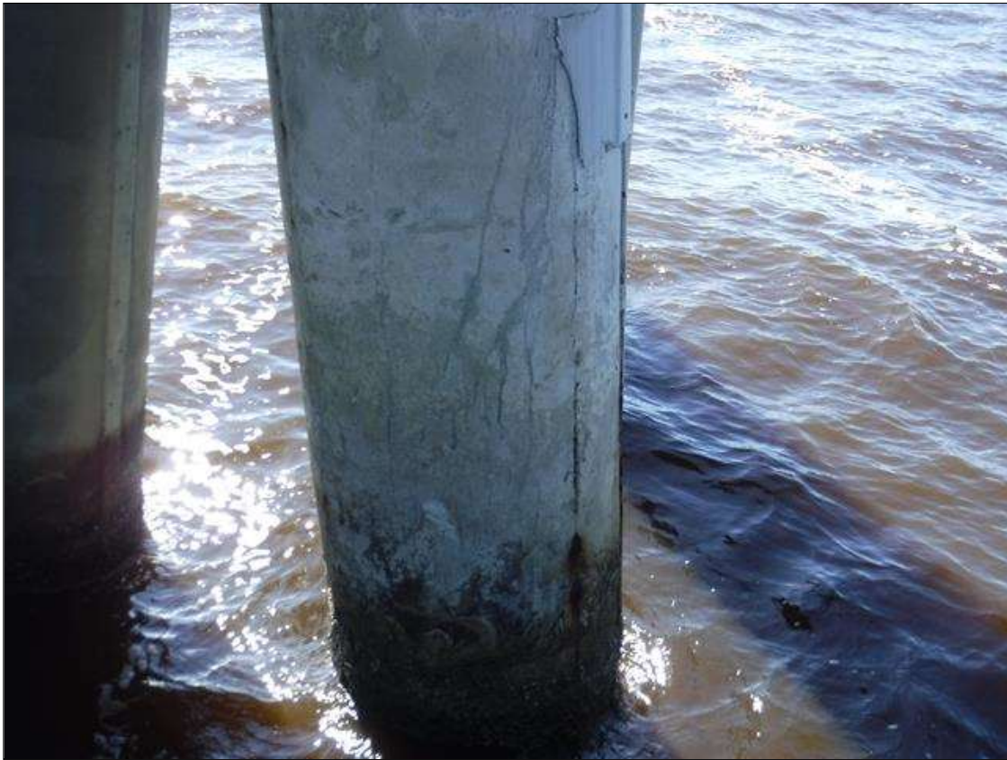
Bent 17 Saved Pile 4: 5' X 1' AREA OF CRACKED DELAMINATION, WITH RUST STAINING, WEST FACE OF PILE JACKET, BEGINNING 4' FROM BOTTOM OF CAP AND EXTENDING BELOW WATERLINE.
