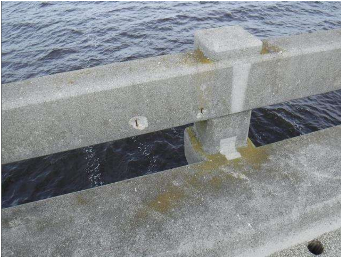
Span 191 Left Bridge Rail: (2) 4" DIAMETER SPALLS WITH EXPOSED REBAR ON RIGHT FACE LOCATED 2' BEFORE POST 2
