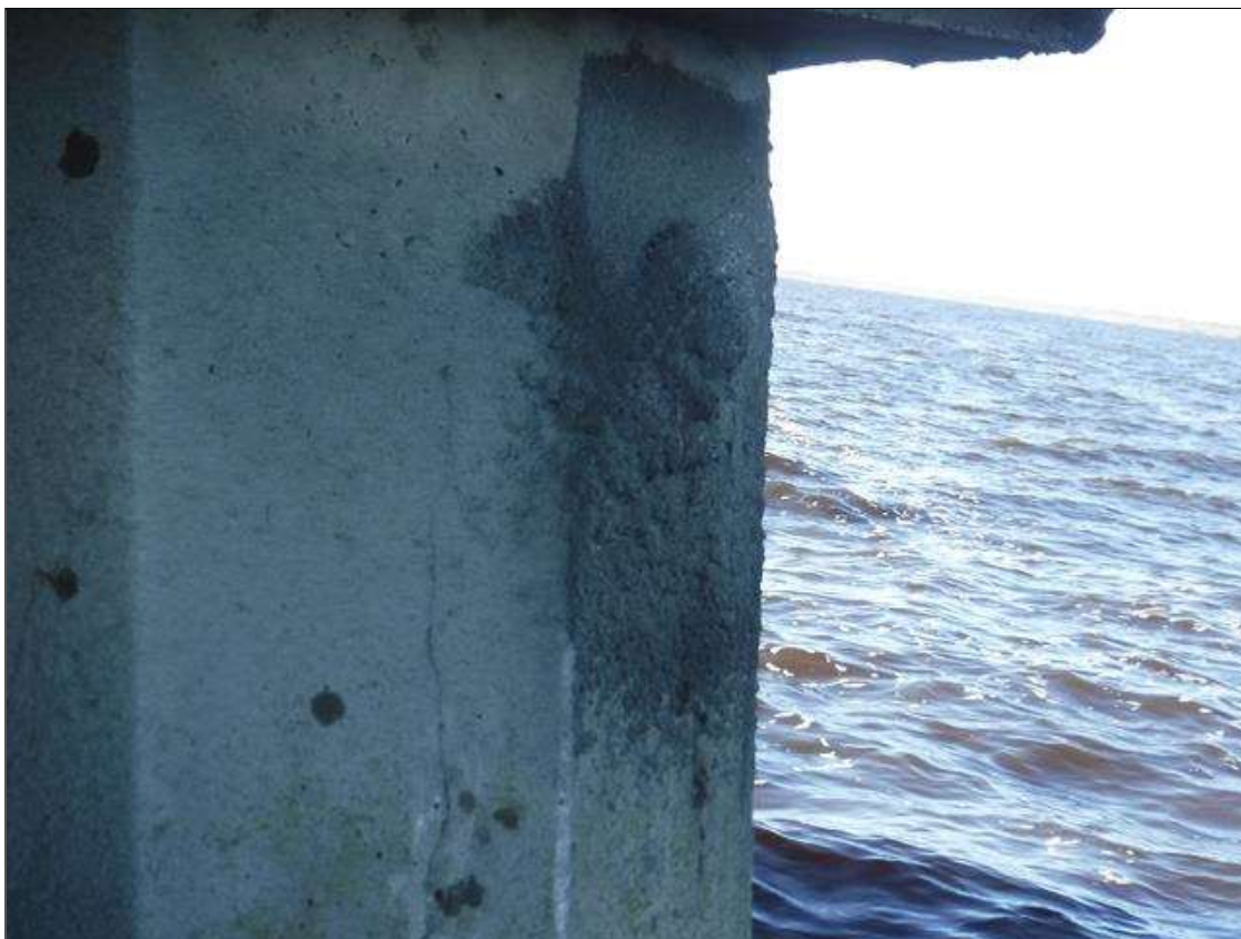
Bent 9 Saved Pile 2: 1' X 1' PATCHED AREA, NORTH FACE, 1' FROM BOTTOM OF CAP.
