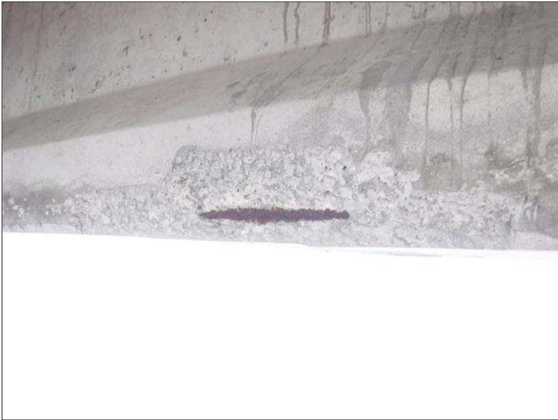
Span 125 Beam 1: (PAR) 2' X 6" X 4" DEEP SPALL WITH EXPOSED STRAND ON SOUTH FACE AT MIDSPAN
