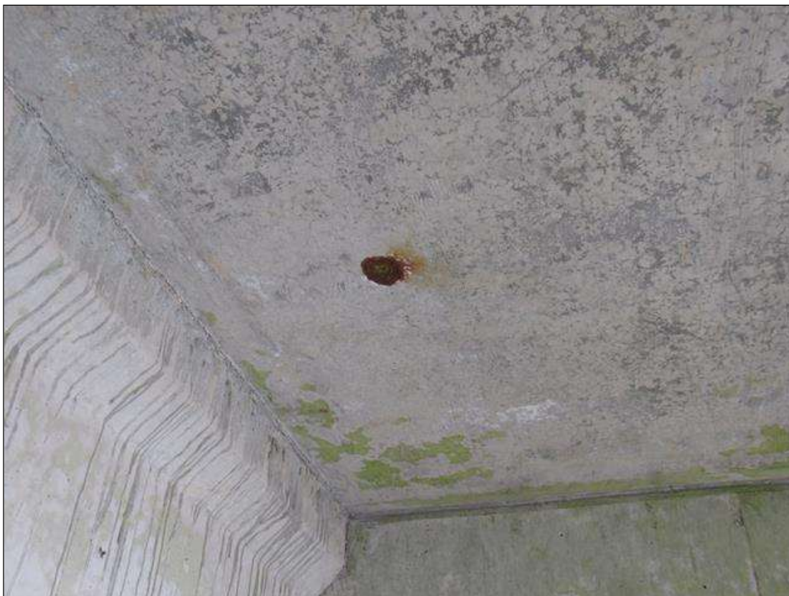
Span 50 Deck: 2" X 2" AREA OF RUST STAINING, UNDERSIDE OF DECK, BETWEEN BEAMS 1 AND 2, 30' FROM BENT 50.
