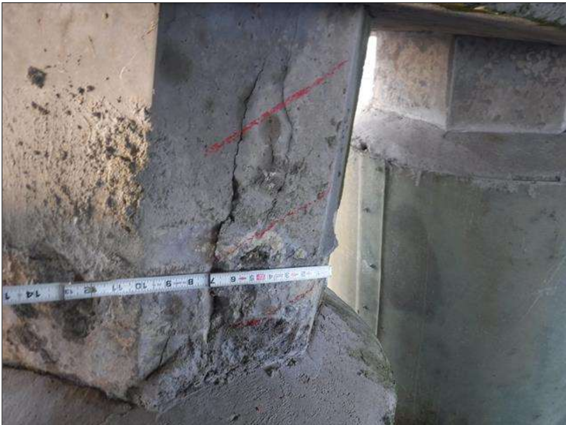
Bent 9 Saved Pile 5: 18" X 8" DELAMINATION ON NORTH FACE BEOW BOTTOM OF CAP, SOUTH FACE SIMILAR
