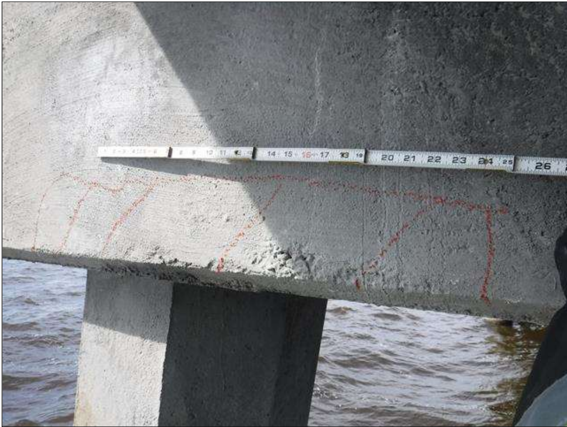
Bent 164 Cap 1: 28" X 6" DELAMINATION IN EAST FACE OVER PILE 4.
