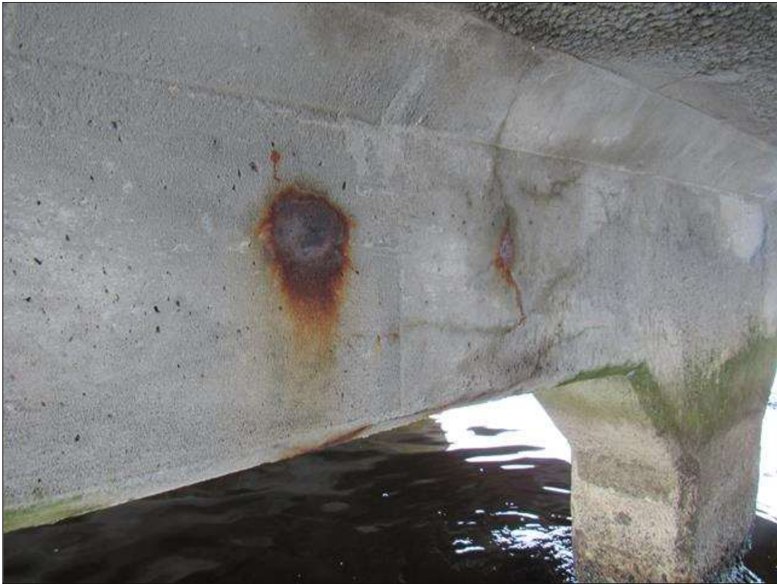
Bent 287 Cap 1: (PAR) 4' OF HAIRLINE TRANSVERSE AND LONGITUDINAL CRACKS, WITH RUST STAINING, AT RANDOM THROUGHOUT EAST FACE.
