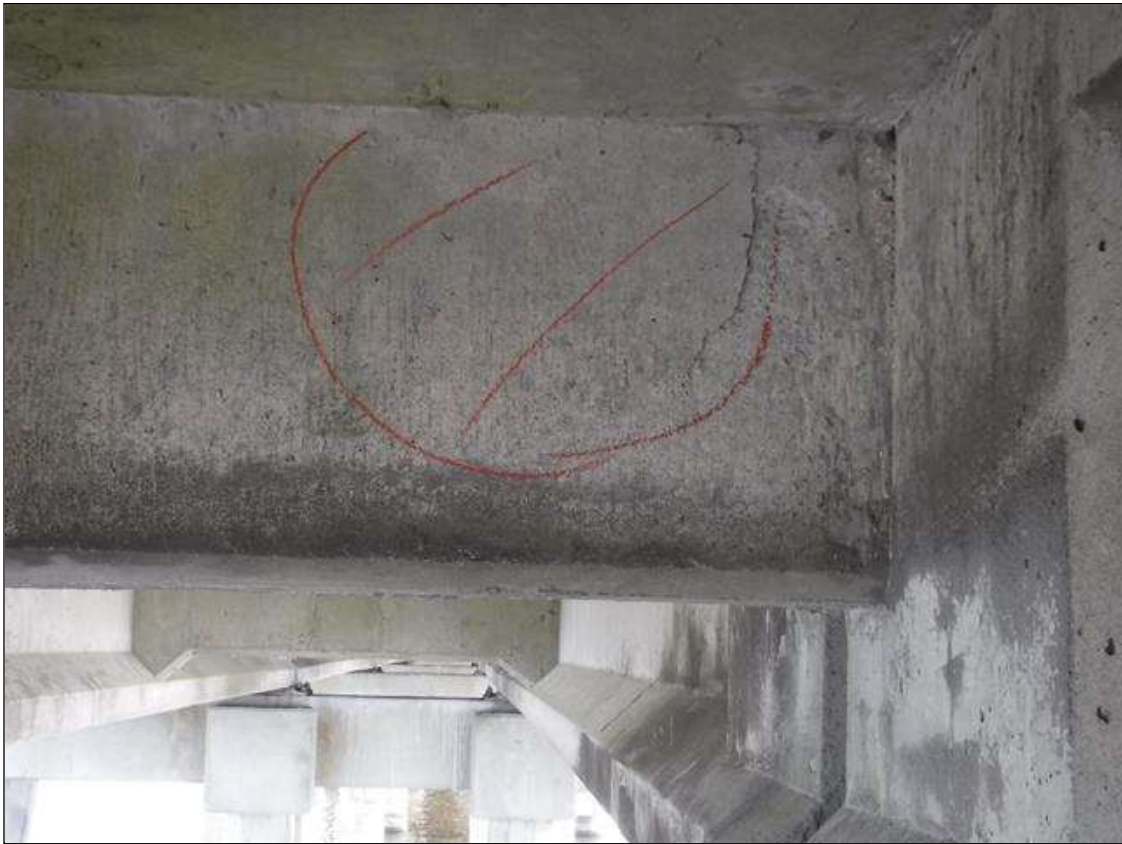
Span 230 Beam 2: 18" DIAMETER DELAMINATION ON END DIAPHRAGM BETWEEN BEAMS 2 AND 3 AT BENT 230
