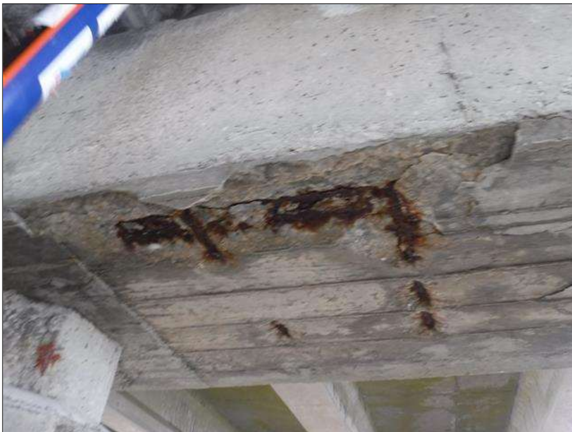
Bent 144 Cap 1: (PAR) 3' X 2" DEEP SPALL IN BOTTOM OF CAP WITH EXPOSED REBAR, REBAR HAS 10% SECTION LOSS
