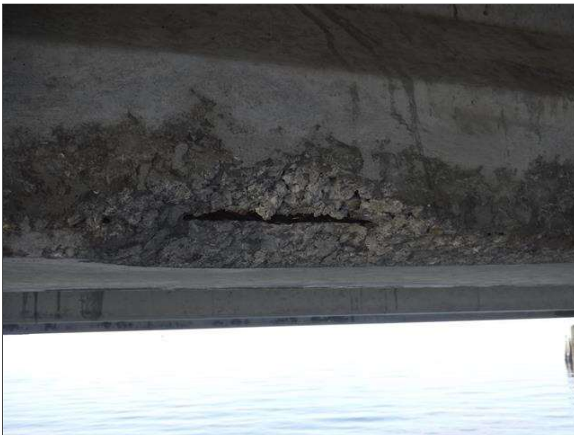
Span 121 Beam 2: (PAR) 20" X 3" X 1" EDGE SPALL, WITH EXPOSED STRAND AND 10 PERCENT SECTION LOSS, BOTTOM NORTH CORNER, 16' FROM BENT 120.
