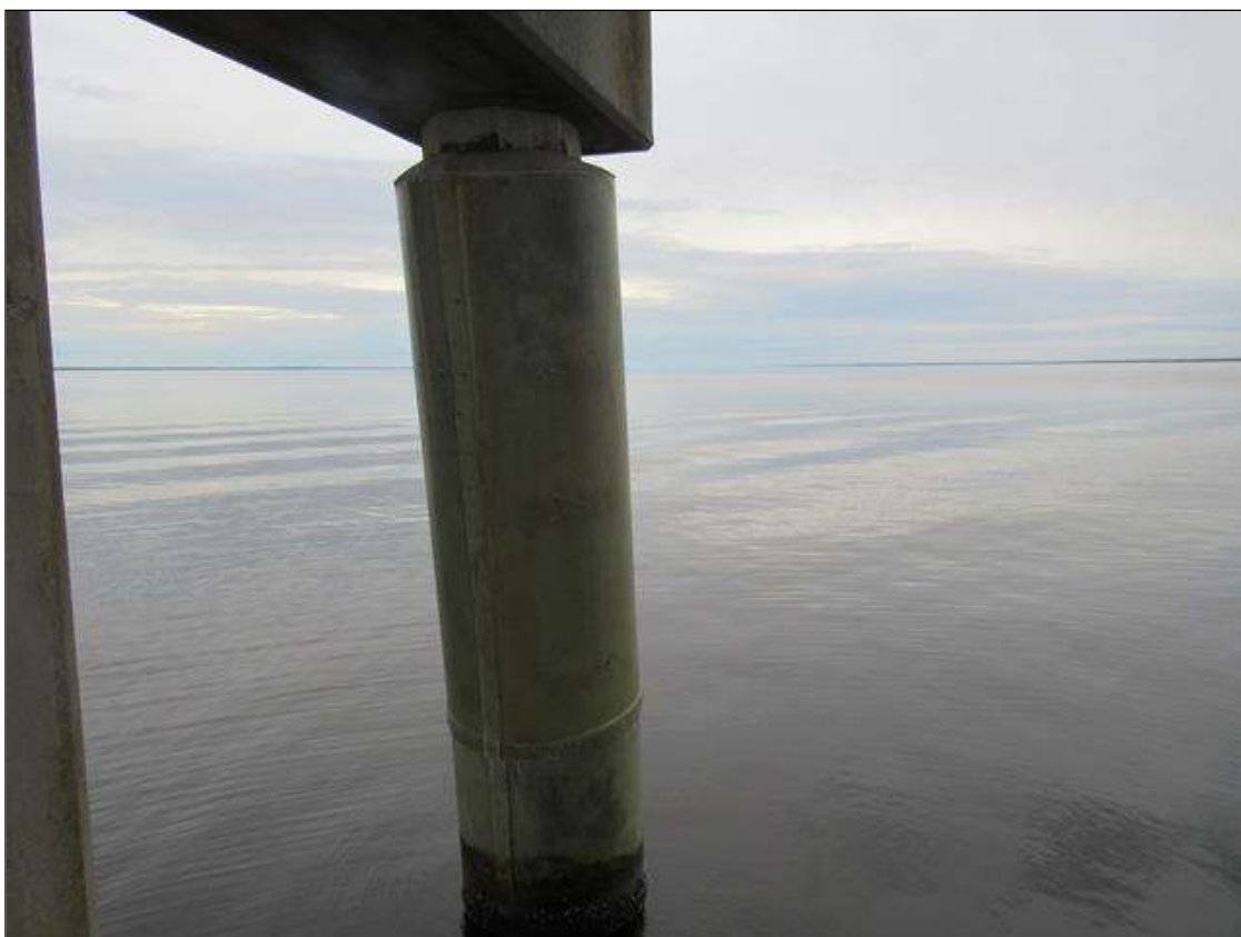
Bent 34 Saved Pile 4: PILE HAS BEEN JACKETED, BEGINNING 1' FROM BOTTOM OF CAP AND EXTENDING BELOW WATERLINE.
