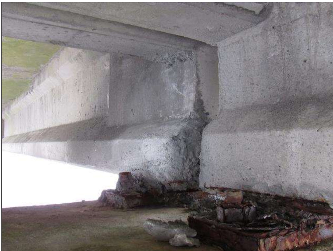
Span 55 Beam 4: 12" X 12" PATCHED AREA, NORTH FACE, AT BENT 54.
