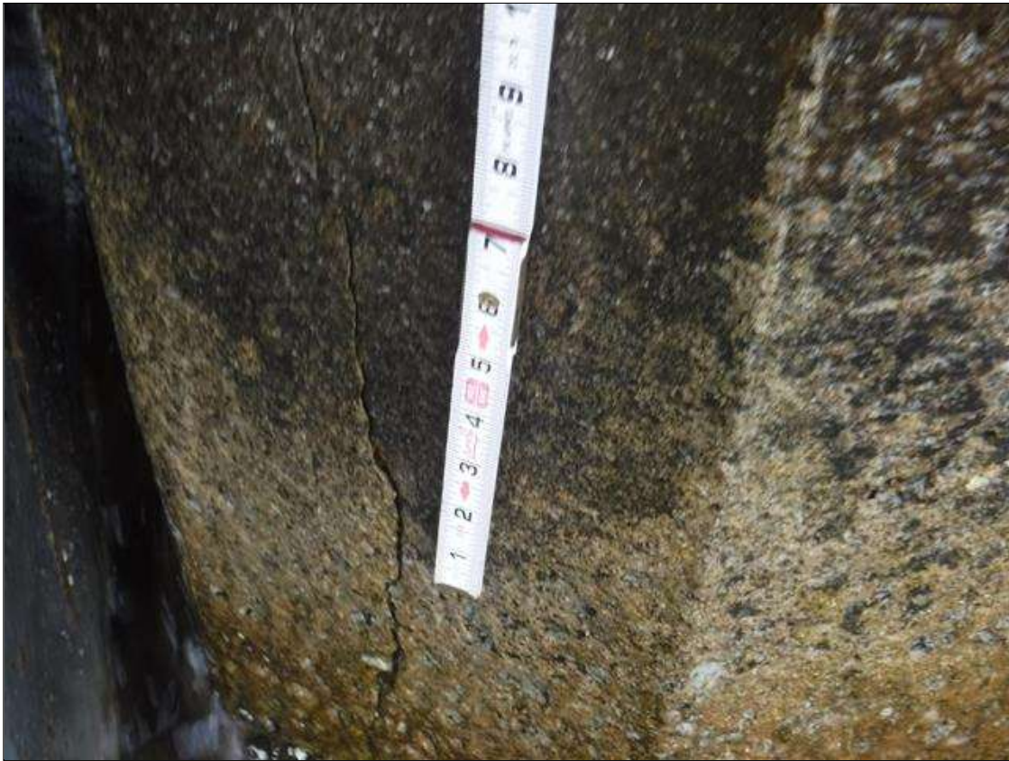
Bent 196 Pile 2: (PAR) 3' LONG X 0.06" WIDE CRACK IN EAST 8' BELOW CAP
