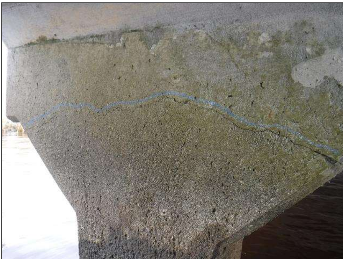
Bent 296 Cap 1: 3' X UP TO 1/16" WIDE LONGITUDINAL CRACK ON WEST FACE LOCATED ABOVE PILE 1
