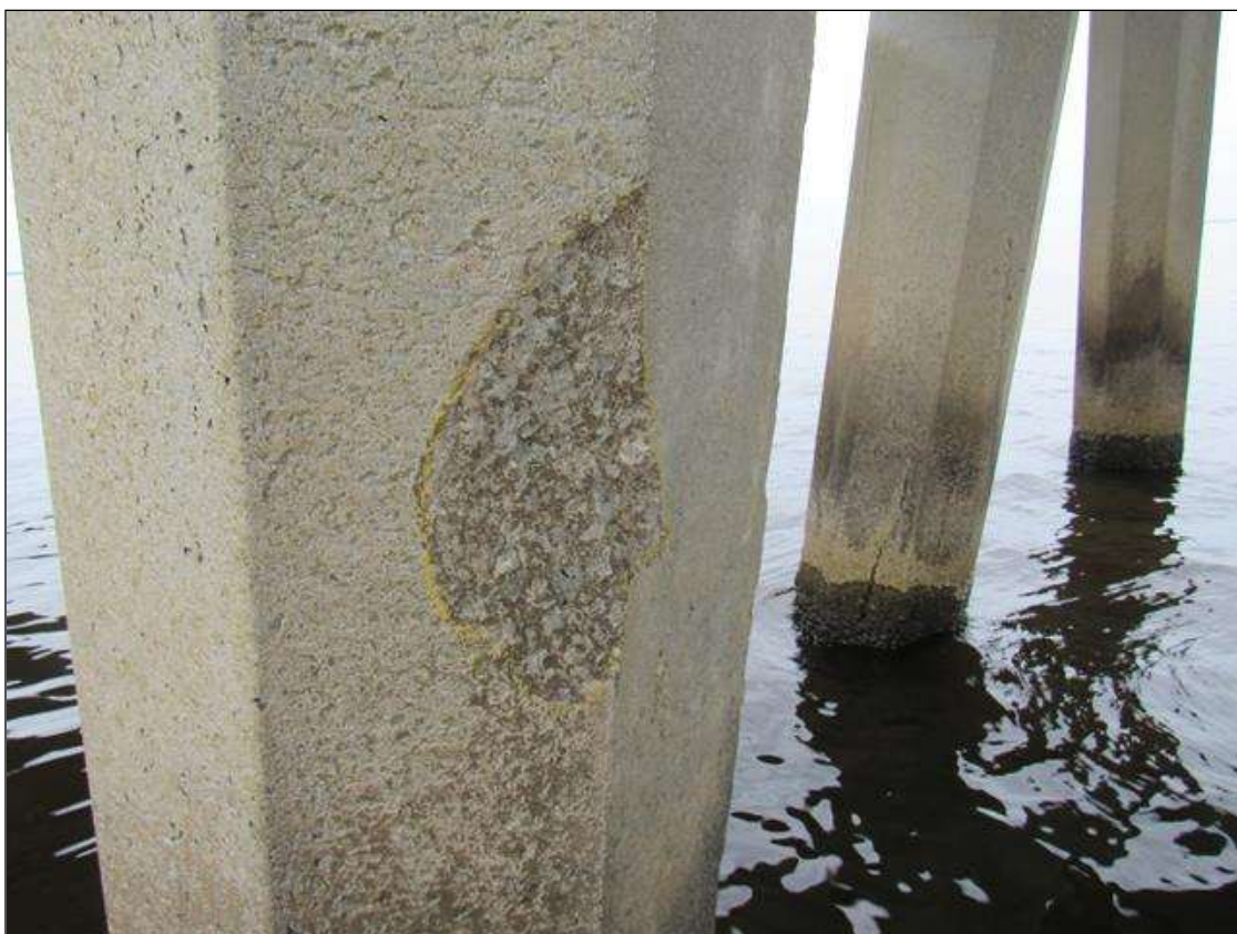
Bent 49 Saved Pile 3: 7" X 14" WIDE X 1.5" DEEP SPALL ON NORTHWEST FACE LOCATED 6' FROM BOTTOM OF CAP
