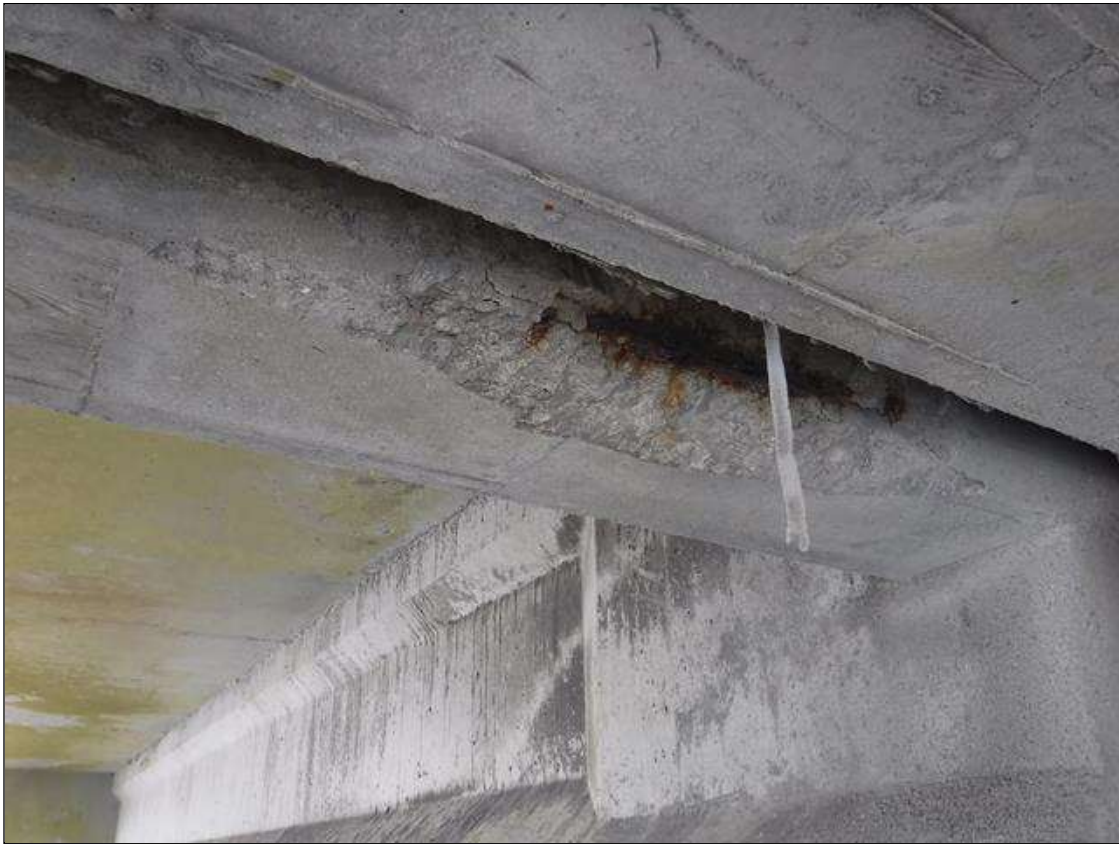
Span 107 Beam 1: (PAR) 2' X 6" X 4" DEEP SPALL WITH EXPOSED REBAR AND 10 PERCENT SECTION LOSS IN BAY 1 DIAPHRAGM AT BENT 106
