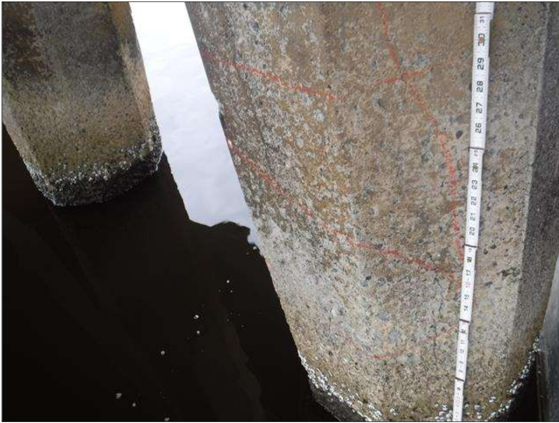
Bent 247 Pile 3: (PAR) (3) UP TO 4' X 0.03" VERTICAL CRACKS ON EAST AND SOUTH FACES WITH 3' X 2' SURROUNDING DELAMINATION ON SOUTH FACE, BEGINNING 6' FROM BOTTOM OF CAP, AT RANDOM THROUGHOUT.
