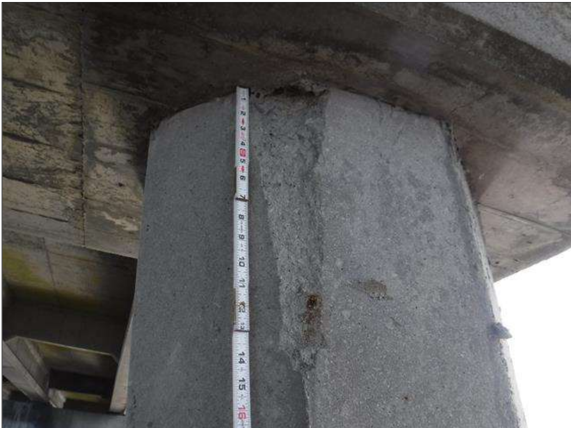
Bent 215 Pile 6: 14" X 4" X 1/2" DEEP SPALL ON WEST FACE BELOW CAP
