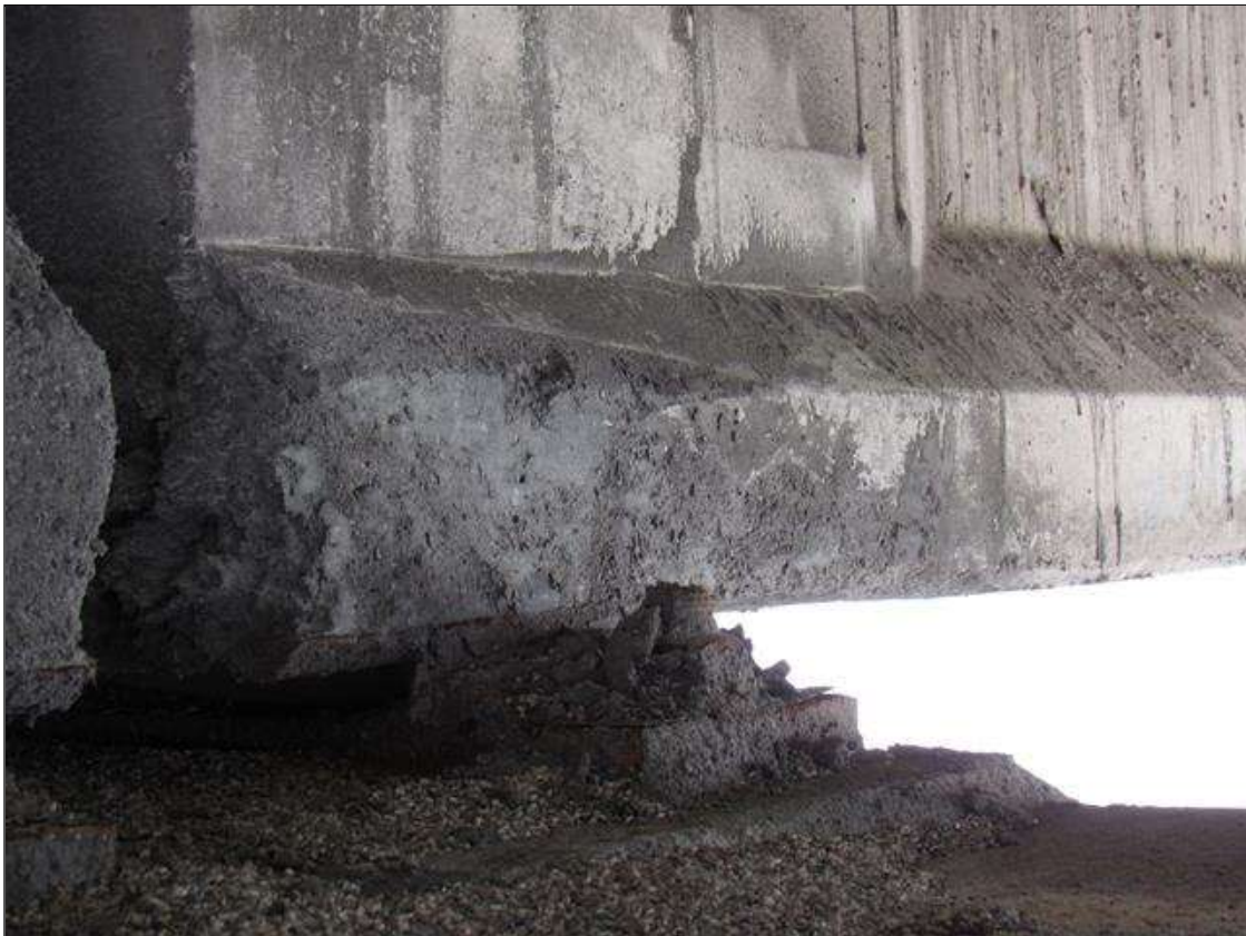
Span 47 Beam 3: 6' X UP TO 18" PATCHED AREA, BOTTOM FACE, EXTENDING 10" ONTO NORTH AND SOUTH FACES, AT BENT 46.
