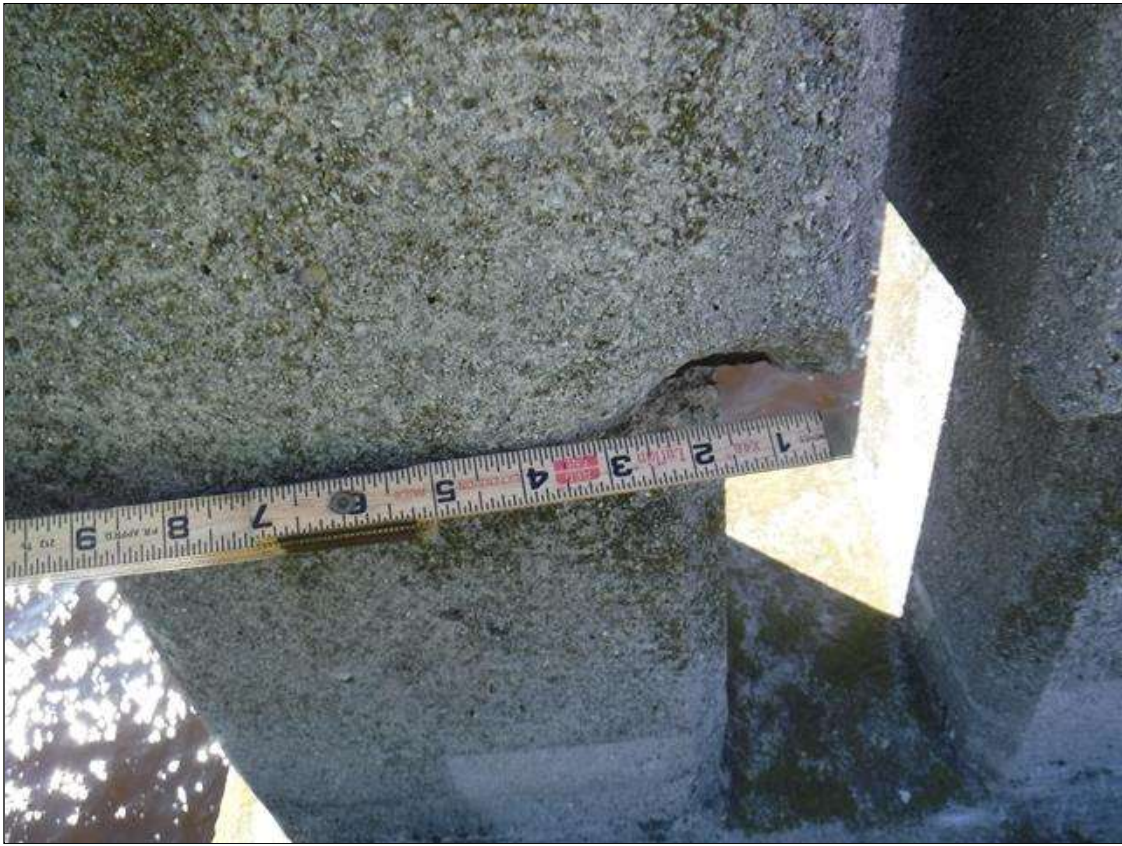
Span 40 Right Bridge Rail: 4" X 3" X 2" SPALL WITH EXPOSED REBAR ON LEFT FACE LOCATED AT 4TH POST FROM BENT 39
