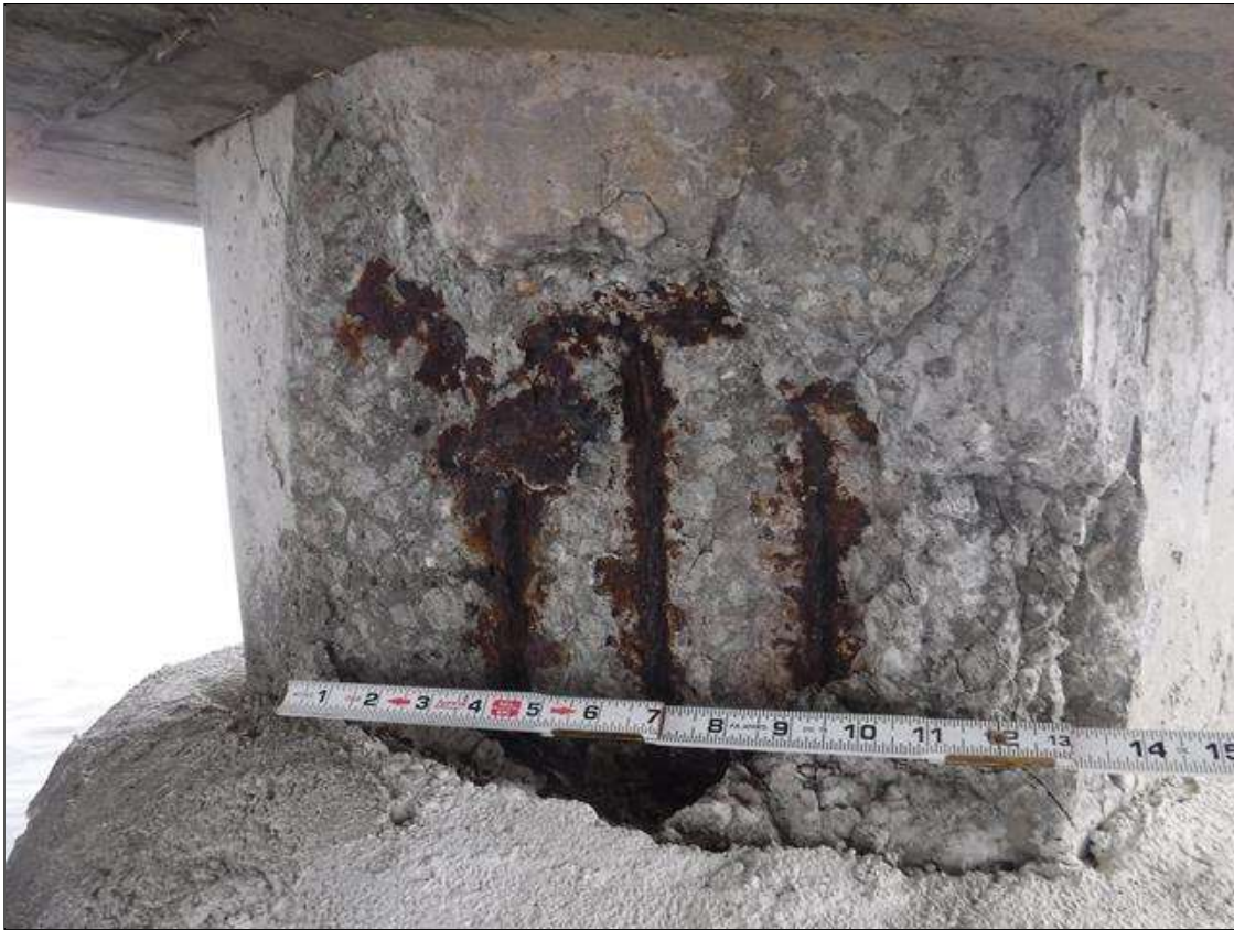
Bent 261 Pile 1: (PAR) 12" X 15" X 3" SPALL, WITH (3) EXPOSED STRAND WITH 50% SECTION LOSS ON SOUTHEAST FACE, AT BOTTOM OF CAP.
