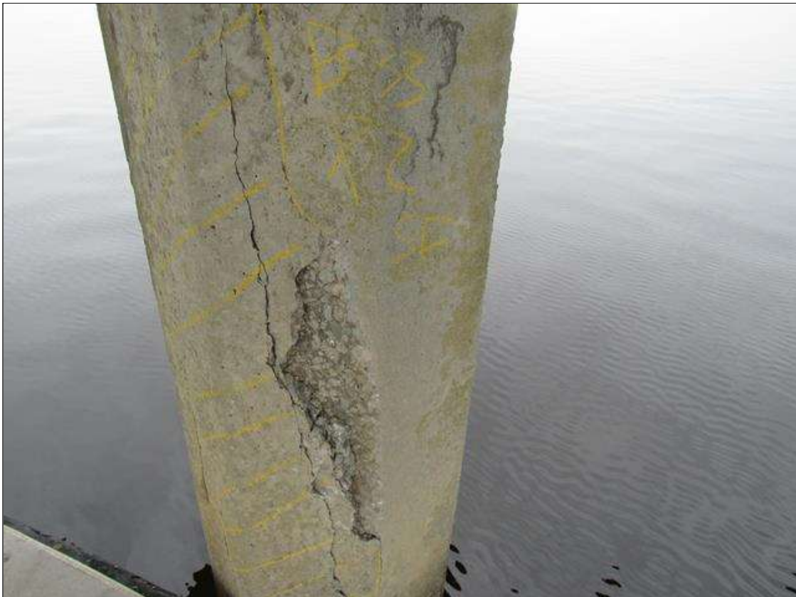
Bent 34 Saved Pile 3: (PAR) 2' X 6" X 1/2" DEEP SPALL WITH 1/16" CRACK, SOUTH FACES, 5' FROM BOTTOM OF CAP.
