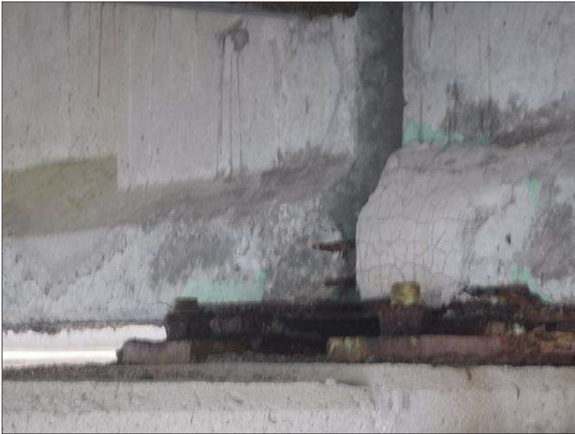
Span 22 Beam 2: (PAR) 6" X 6" X 3" SPALL, WITH EXPOSED PRESTRESSING STRAND, NORTH FACE, AT BENT 21.
