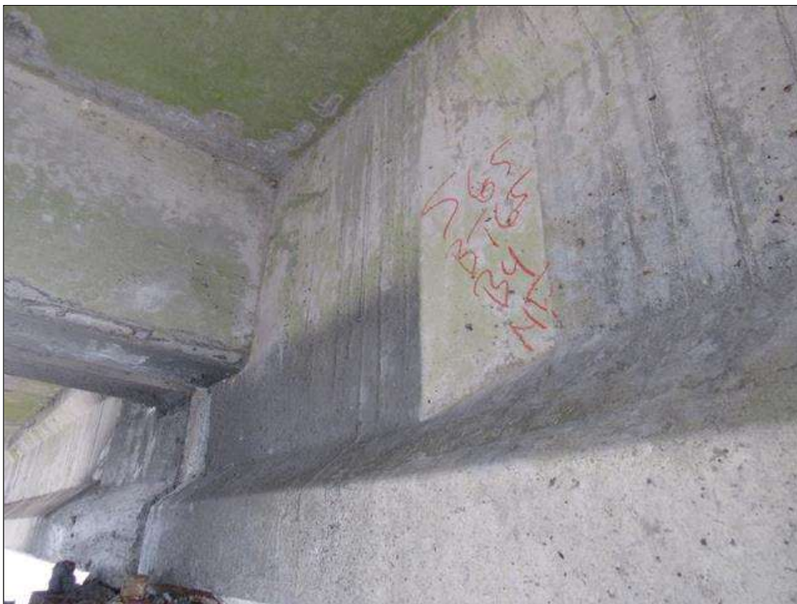
Span 65 Beam 4: 36" X UP TO 36" PATCHED AREA, WITH 3" X 2" X UP TO 1" SPALL, NORTH FACE, AT BENT 65. DEFECT NOT OBSERVED IN 2020 INSPECTION.
