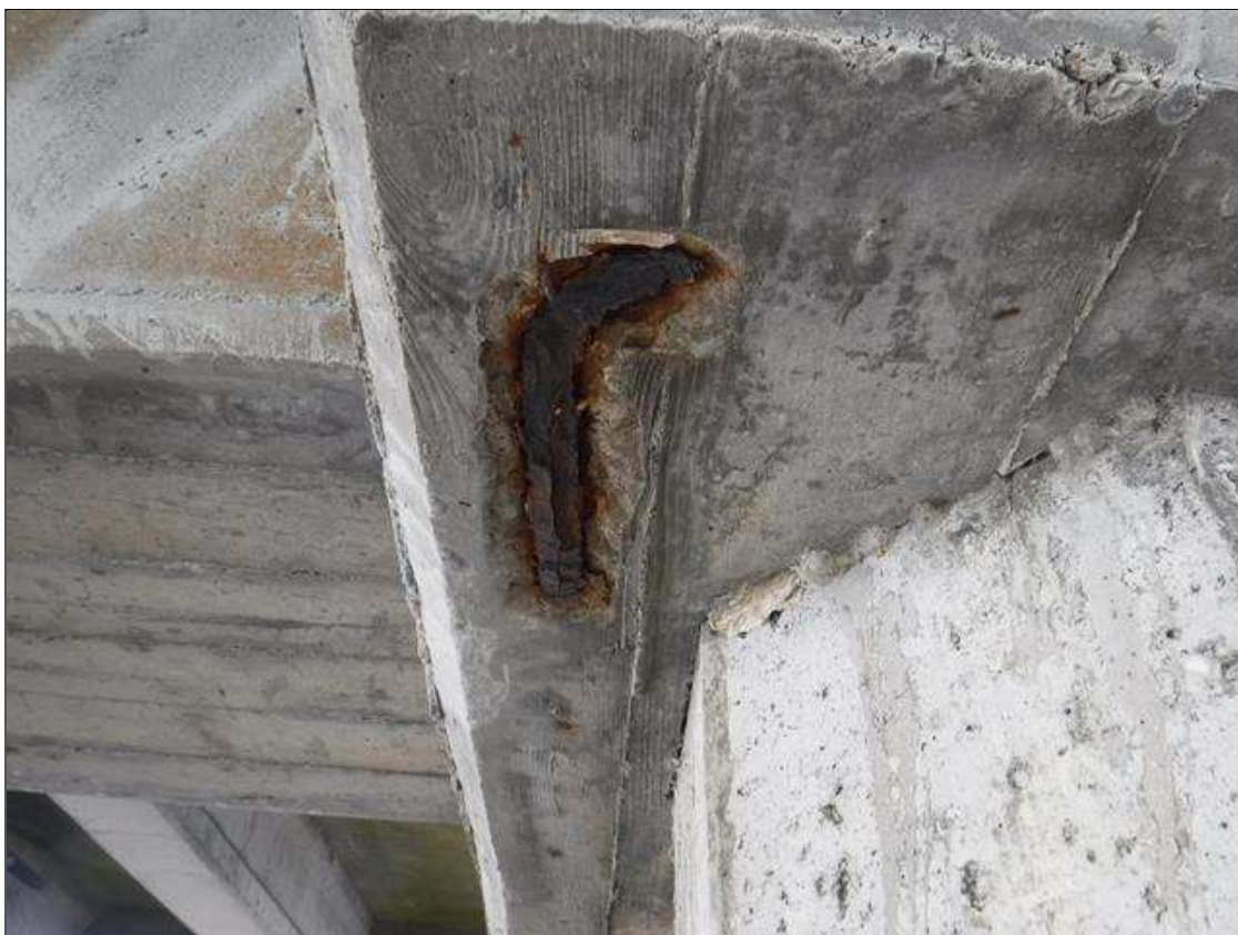
Bent 231 Cap 1: 3' X 8" X 3/4" SPALL, WITH EXPOSED REINFORCING, BOTTOM FACE, BENEATH BEAM 2.
