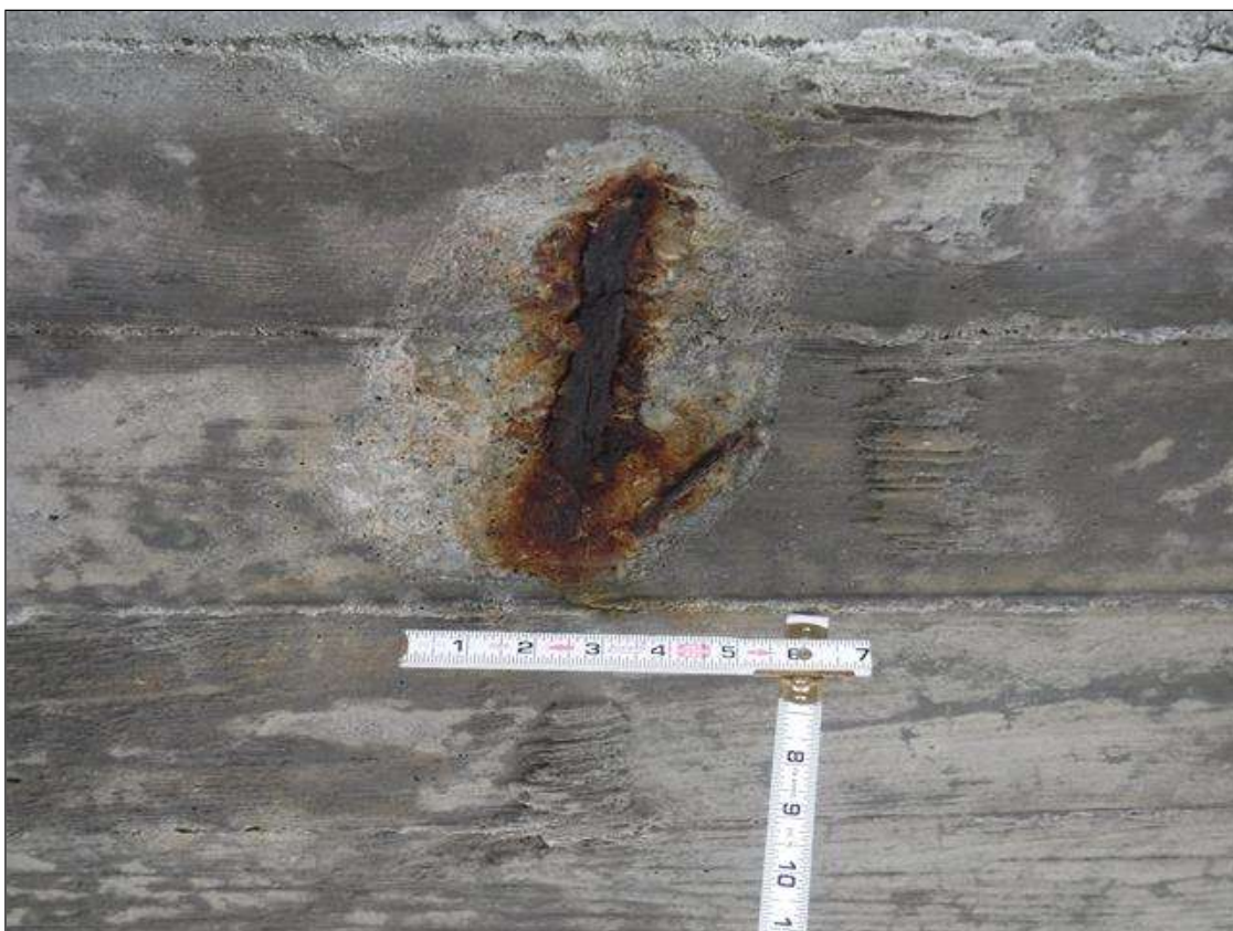
Bent 179 Cap 1: 8" X 5" X 1/4" SPALL, WITH EXPOSED REINFORCING, BOTTOM FACE, AT MID SPAN.
