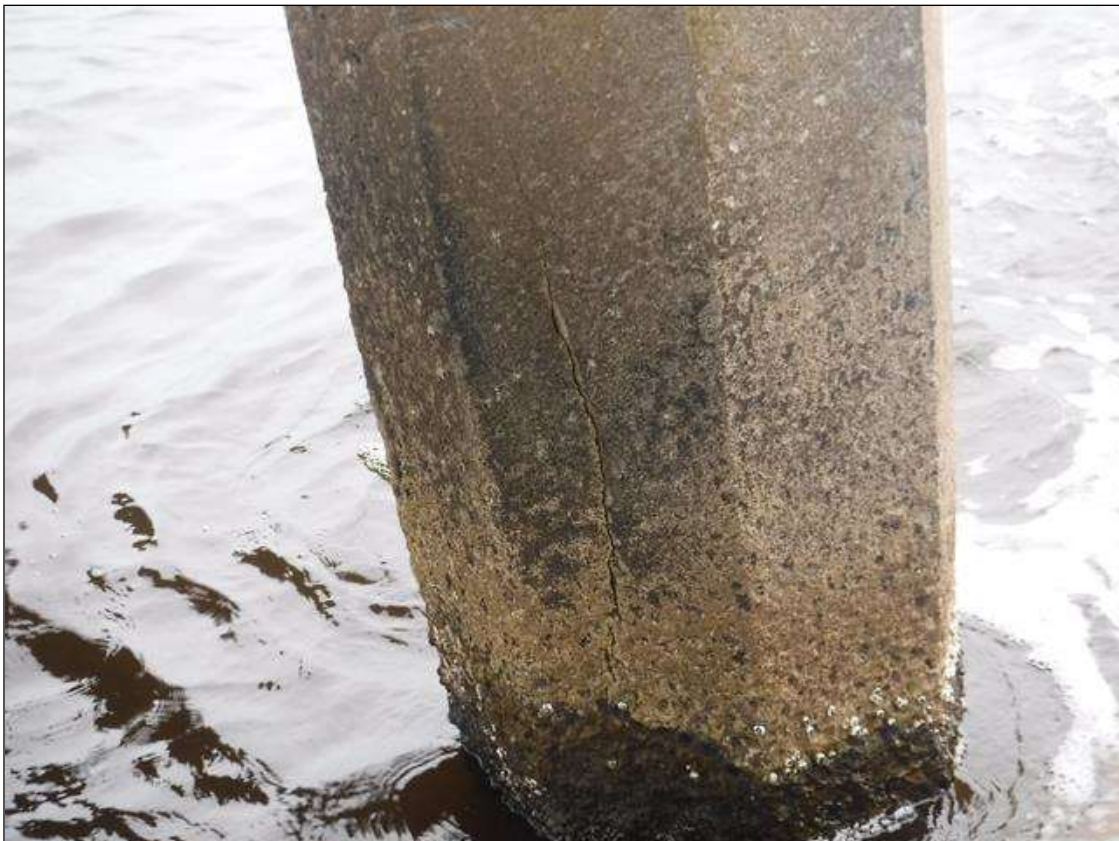
Bent 252 Pile 4: (PAR) (2) UP TO 2' X 0.016" VERTICAL CRACKS, NORTH FACE, 8' FROM BOTTOM OF CAP, WITH ADJACENT 2' X 1' DELAMINATION.
