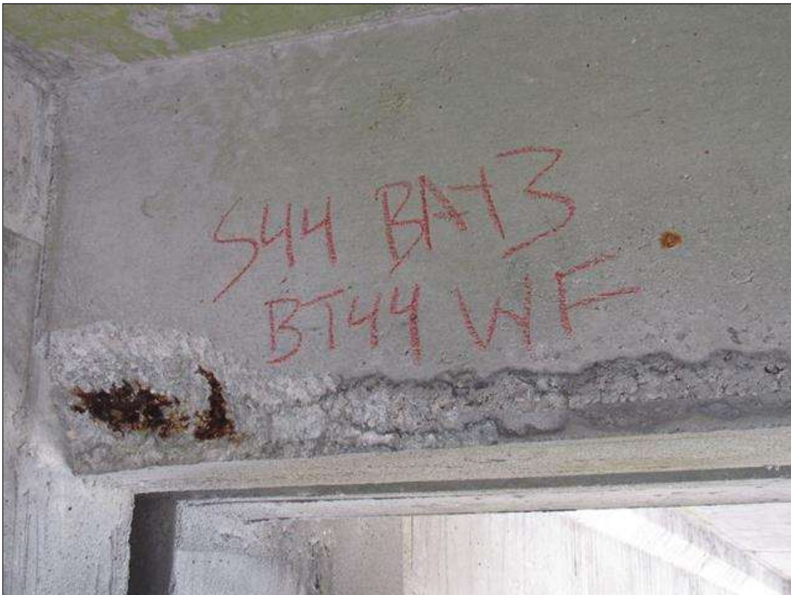
Span 44 Beam 3: 20" X 6" X 4" DEEP SPALL WITH EXPOSED REBAR ON END DIAPHRAGM IN BAY 3, AT BENT 44
