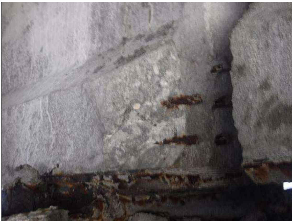
Span 161 Beam 3: (PAR) 10" X 10" X 1" DEEP SPALL WITH EXPOSED STRAND ON SOUTH FACE AT BENT 161
