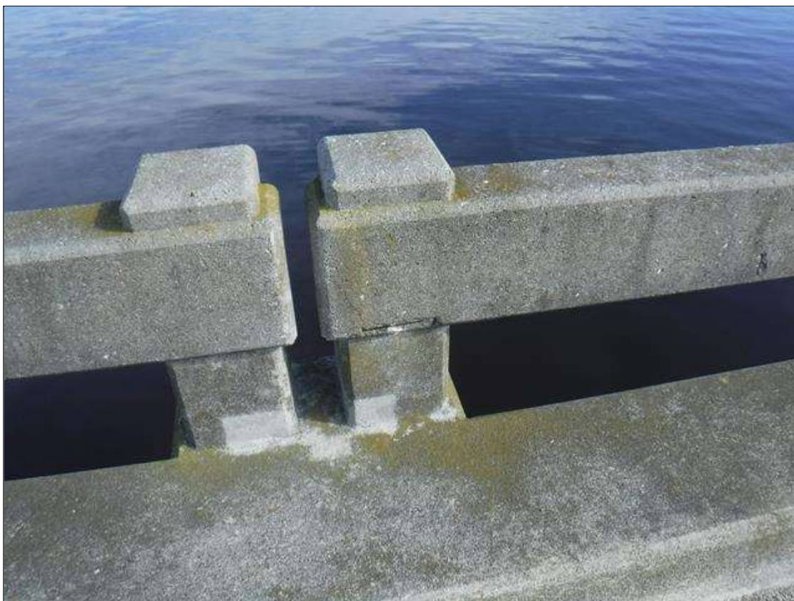
Span 269 Left Bridge Rail: 7" X 2" X 1" DEEP SPALL WITH EXPOSED REBAR ON RIGHT FACE ON POST 7
