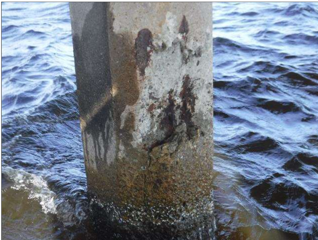
Bent 123 Pile 5: (PAR) 28" X 20" X 2" SPALL WITH EXPOSED STRAND, SOUTH FACE, 8' FROM BOTTOM OF CAP.
