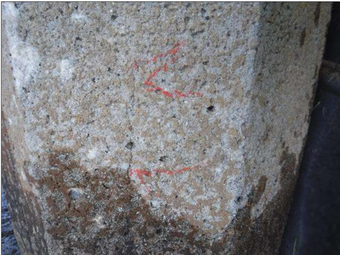
Bent 162 Pile 4: (PAR) HAIRLINE TO 1/16" CRACKS, 6' BELOW CAP, DOWN 10', MULTIPLE FACES. SCALING TO 1" DEEP WITH LOOSE AGGREGATE FROM WATERLINE TO MUDLINE.
