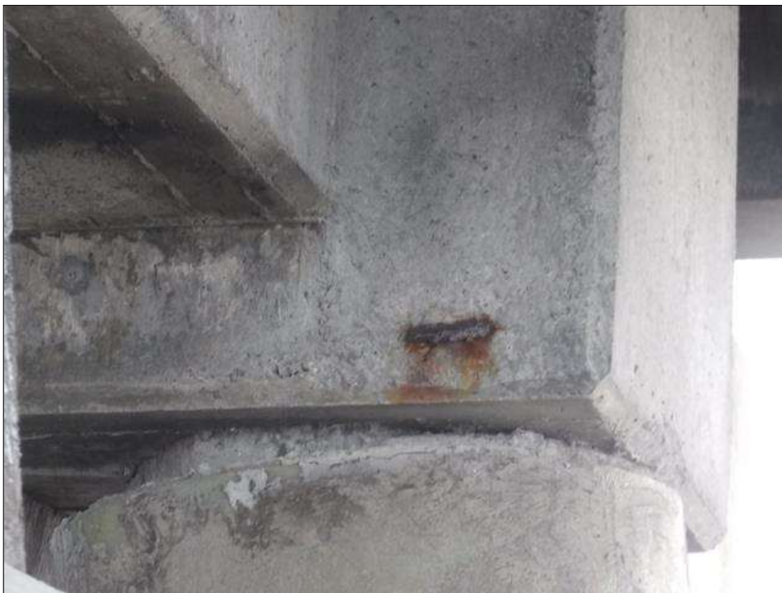
Bent 147 Cap 1: 8" X 4" X 1" SPALL, WITH EXPOSED REINFORCING, NORTH FACE OF PILE 4 BLOCK-OUT.
