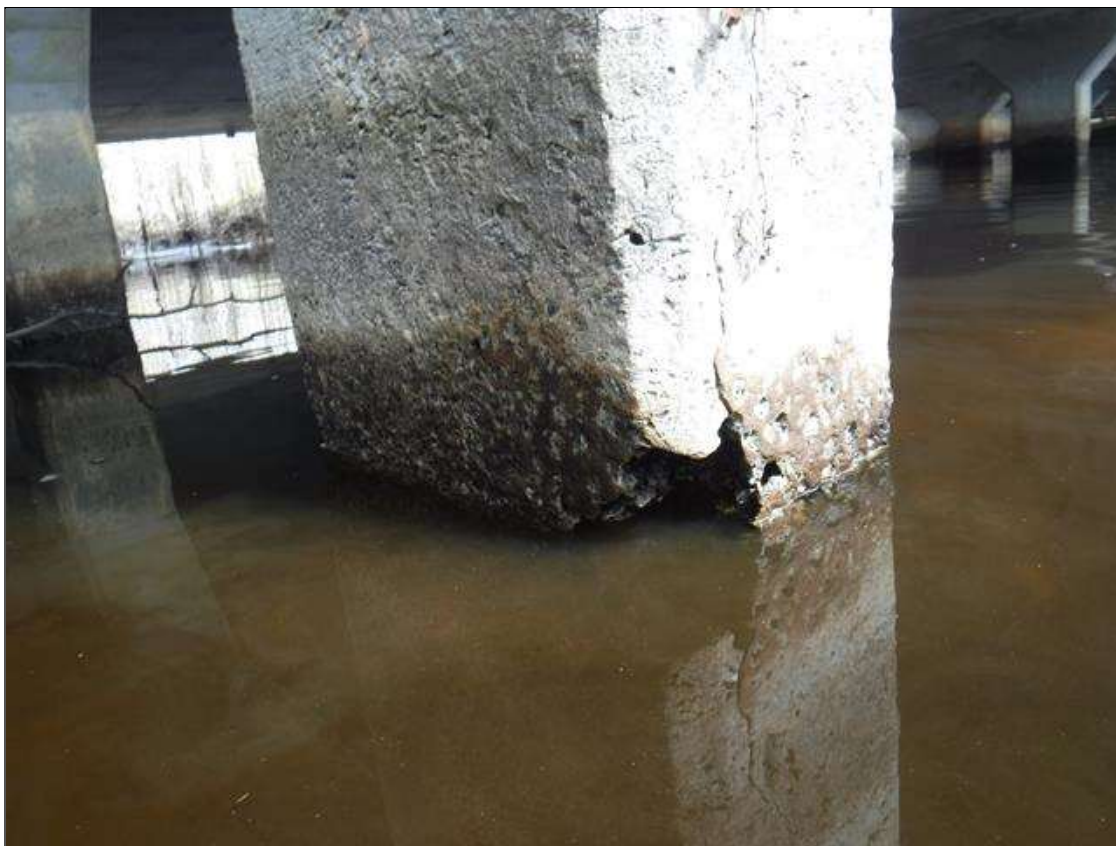
Bent 308 Pile 4: 12" X 8" X 8" SPALL AT BOTTOM EAST CORNER
