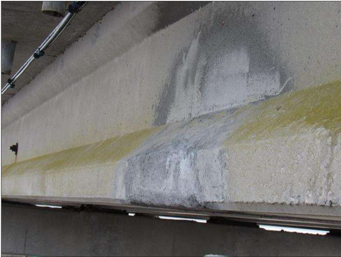
Span 47 Beam 1: 4' X UP TO 5" PATCHED AREA, BOTTOM FACE, EXTENDING 12" ONTO NORTH FACE, 6' FROM BENT 46.
