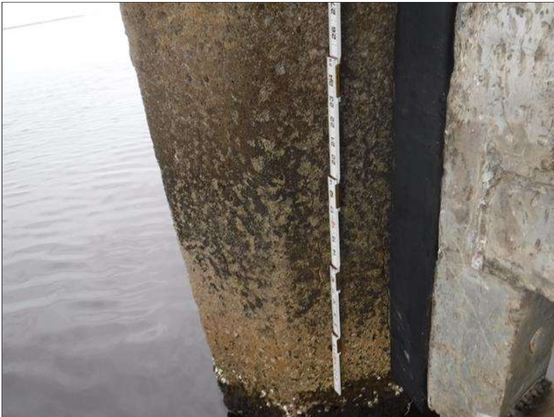
Bent 249 Pile 4: (PAR) (2) UP TO 3' X 0.03" VERTICAL CRACKS ON NORTH FACE, BEGINNING 7' BOTTOM OF CAP
