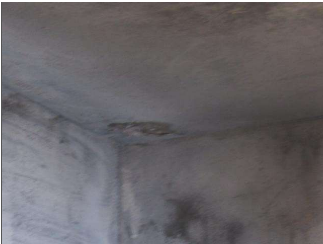
Span 4 Deck: 8" X 8" X 1" SPALL, DECK UNDERSIDE, BETWEEN BEAMS 2 AND 3, AT BENT 3.
