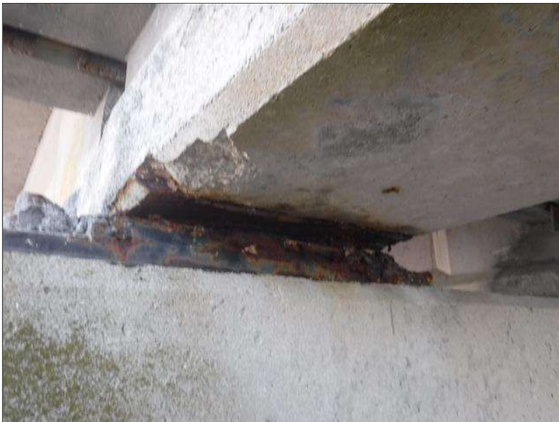
Span 72 Beam 1: 6" X UP TO 5" X 1.5" DEEP SPALL, BOTTOM FACE, AT BENT 72.
