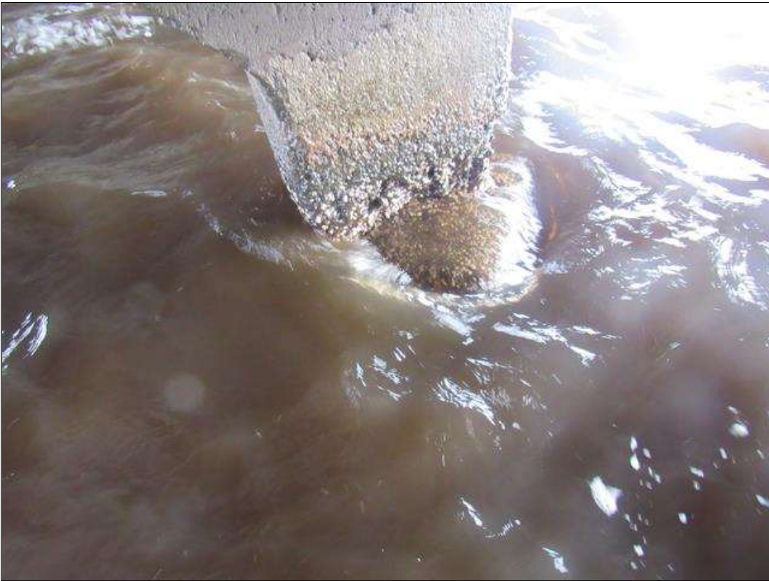
Bent 292 Pile 3: (PAR) 6" X 20" X 6" SPALL, WITH EXPOSED PRIMARY REBAR, WEST FACE, 2' FROM BOTTOM OF CAP. REBAR HAS 10% SECTION LOSS
