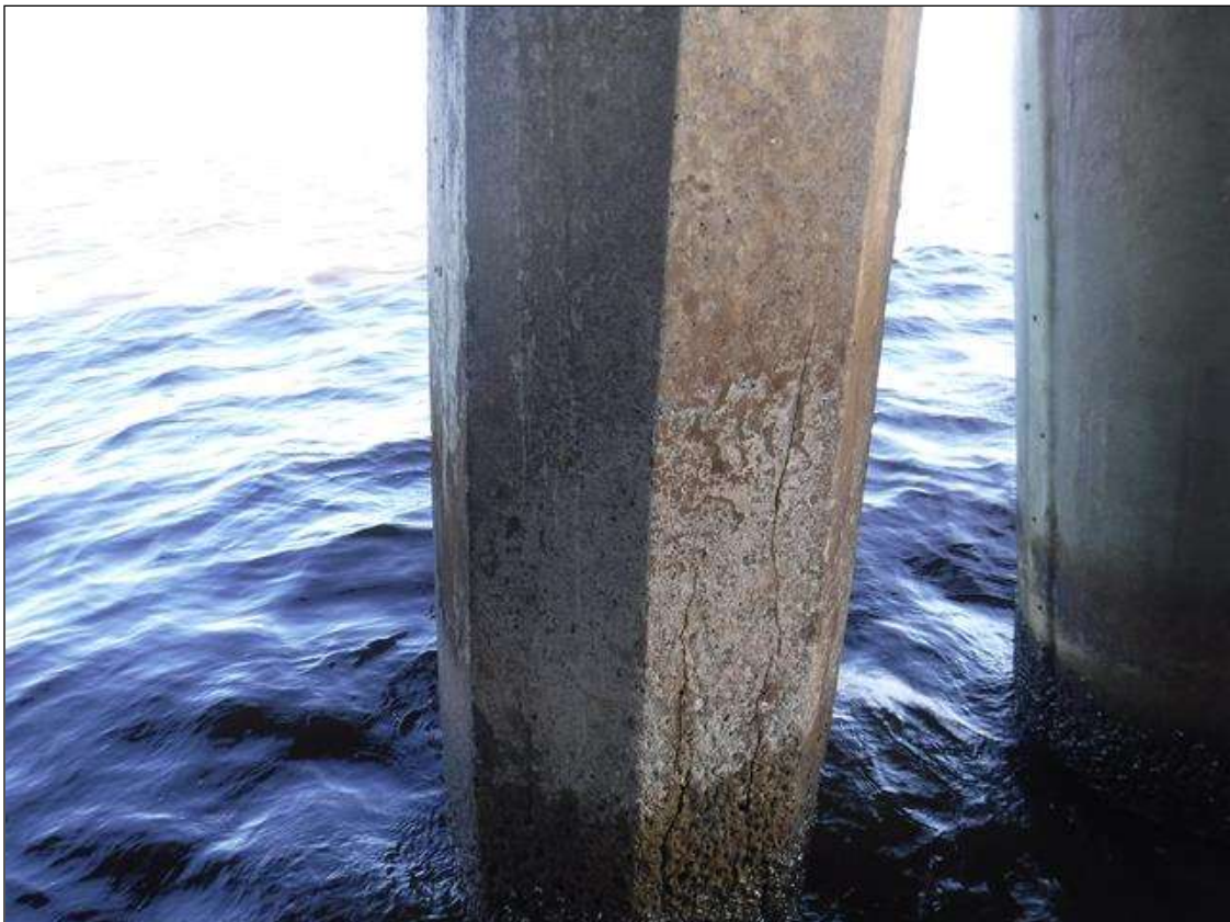
Bent 9 Saved Pile 2: (PAR) HAIRLINE TO 1/16" CRACKS, 3' BELOW CAP, DOWN 4', MULTIPLE FACES. SCALING TO 1" DEEP FROM WATERLINE TO MUDLINE.
