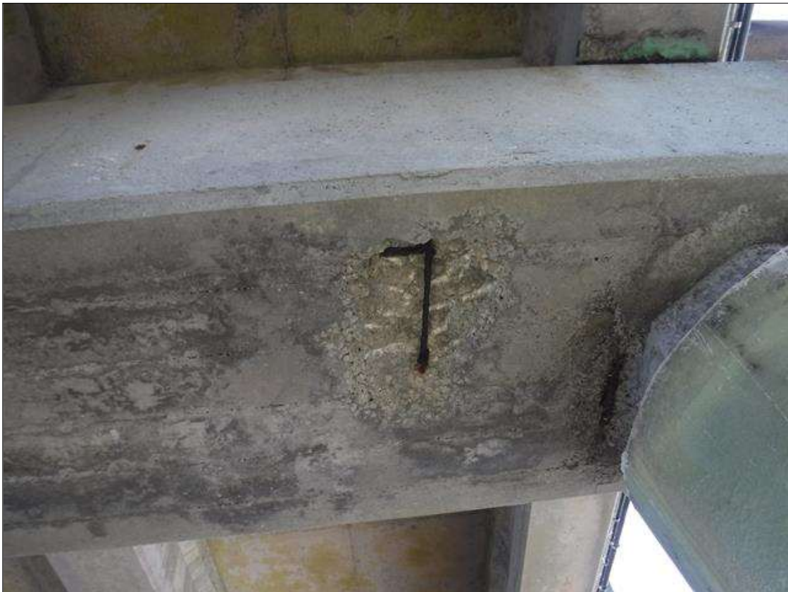
Bent 22 Cap 1: (PAR) 12" X 24" X 6" SPALL, WITH EXPOSED PRIMARY REINFORCING, BOTTOM FACE, BETWEEN BEAMS 3 AND 4. REBAR HAS 10% SECTION LOSS
