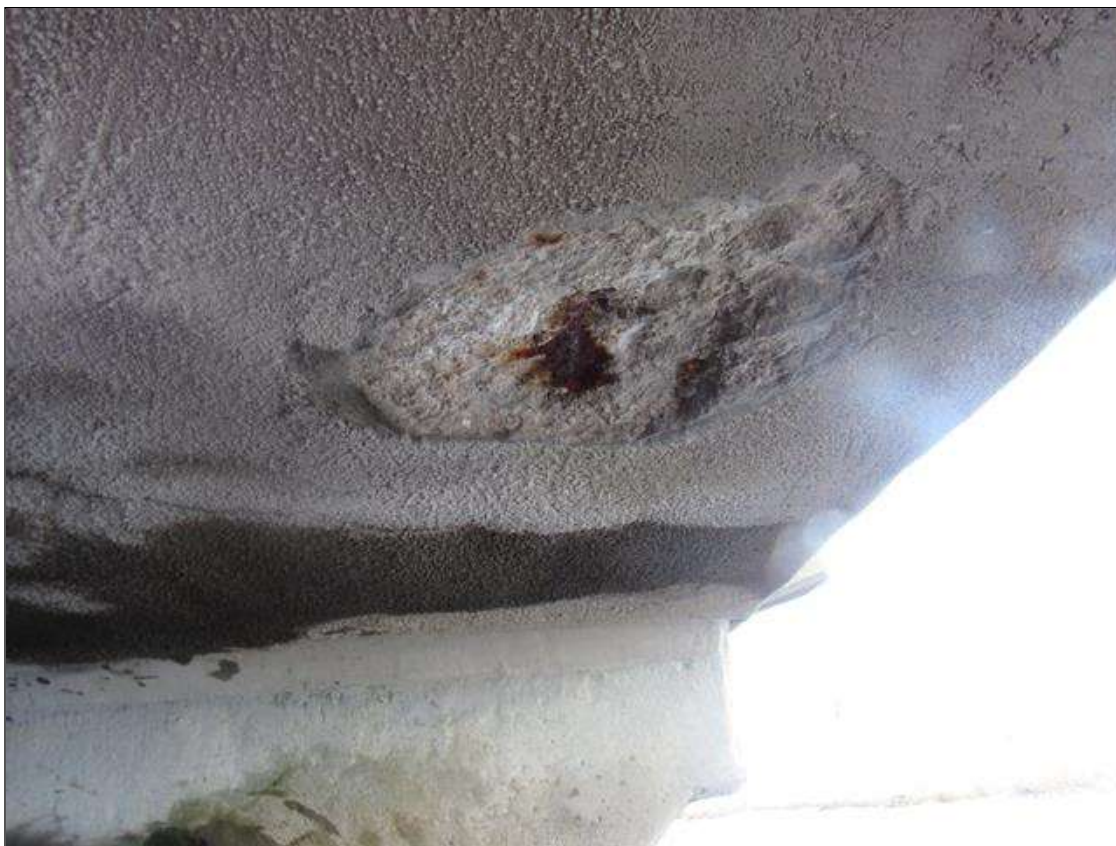
Span 294 Deck: 16" DIAMETER X 2" SPALL, WITH EXPOSED REINFORCING, DECK UNDERSIDE, 2' FROM SOUTH FACE, NEAR MIDSPAN.
