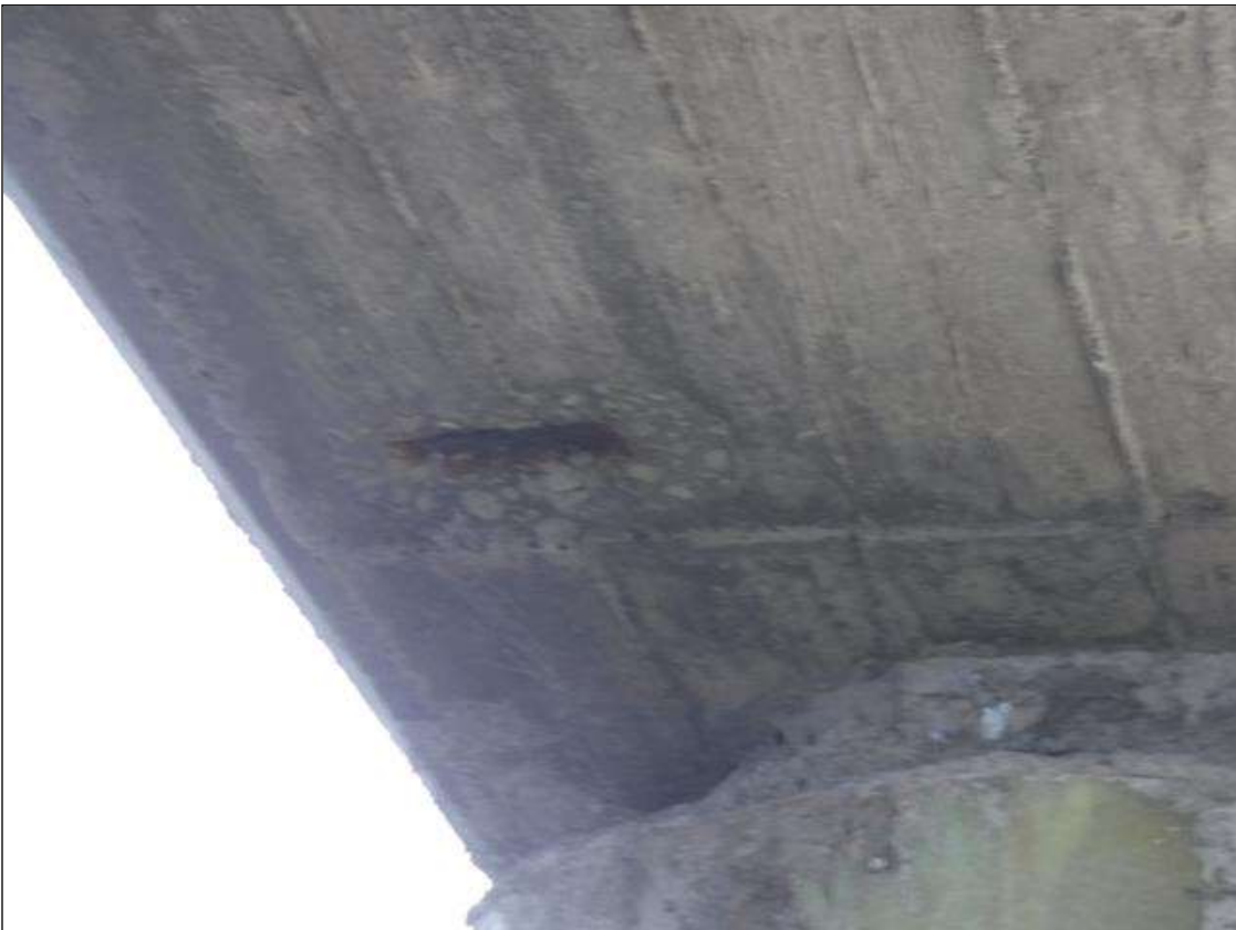
Bent 128 Cap 1: 8" X 4" X 1/2" SPALL, WITH EXPOSED REINFORCING, BOTTOM FACE, NEAR PILE 4.
