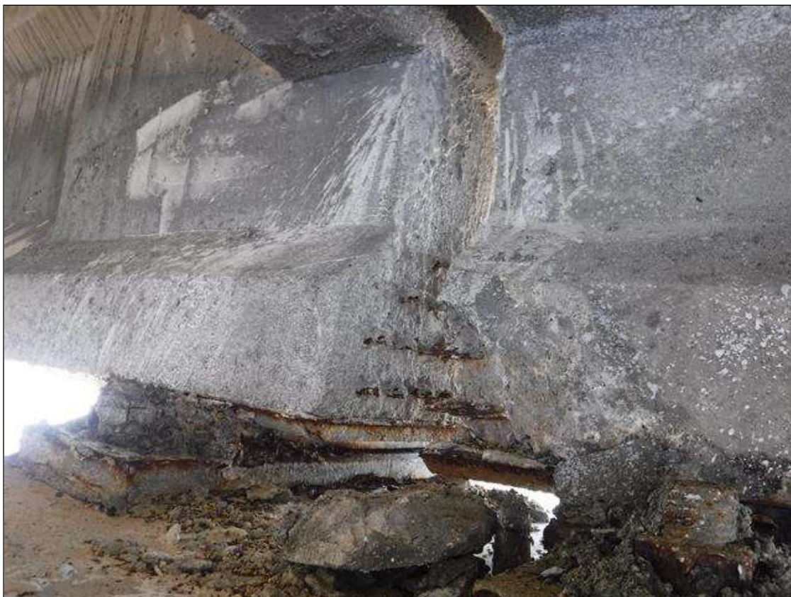
Span 138 Beam 4: (PAR) 6" X 6" X 2" DEEP SPALL WITH EXPOSED STRAND ON NORTH FACE AT BENT 138
