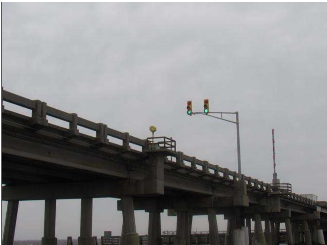
UTILITIES ATTACHED TO RIGHT SIDE OF BENTS 108, 109, AND 110
