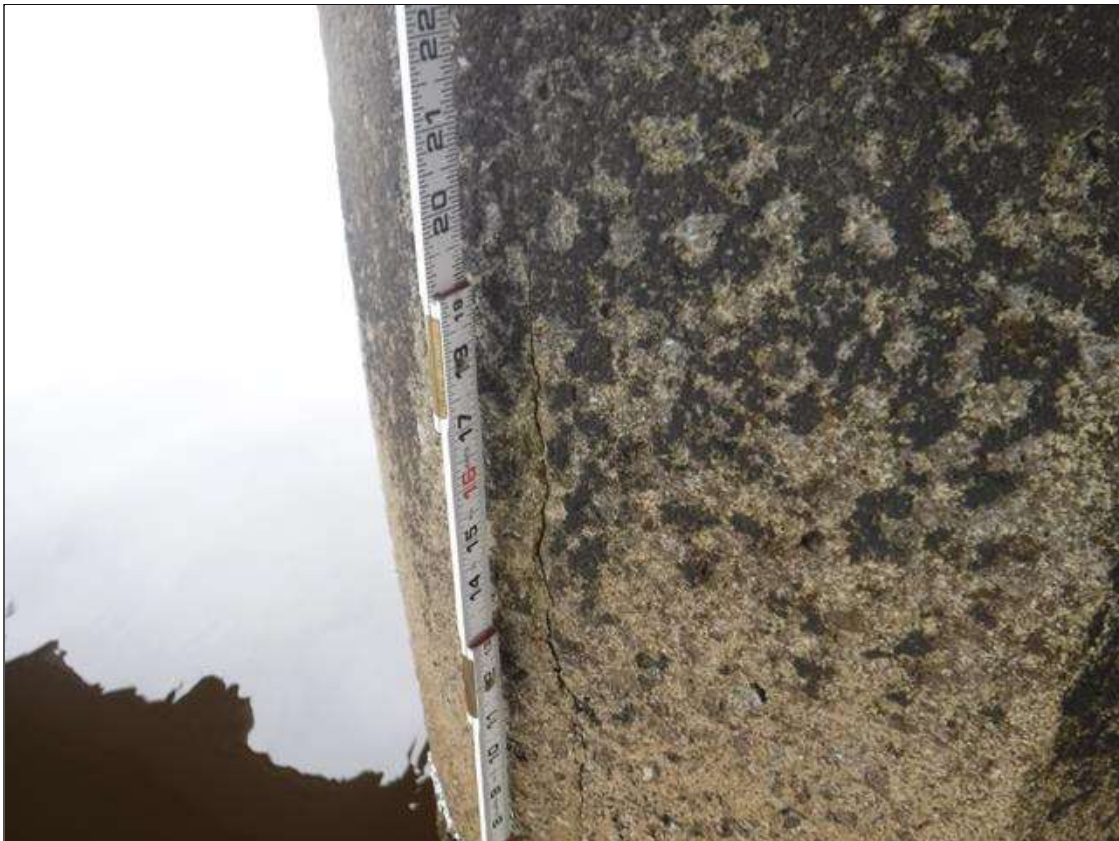
Bent 233 Pile 3: (PAR) (3) UP TO 4' X 0.03" VERTICAL CRACKS, BEGINNING 6' FROM BOTTOM OF CAP, AT RANDOM THROUGHOUT. WITH 2' X 1' ADJACENT DELAMINATION ON NORTH FACE
