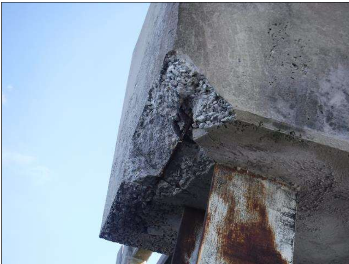
Bent 120 Cap 1: 24" X 8" X 8" EDGE SPALL, WITH EXPOSED PRIMARY REINFORCING, BOTTOM OF NORTH FACE.
