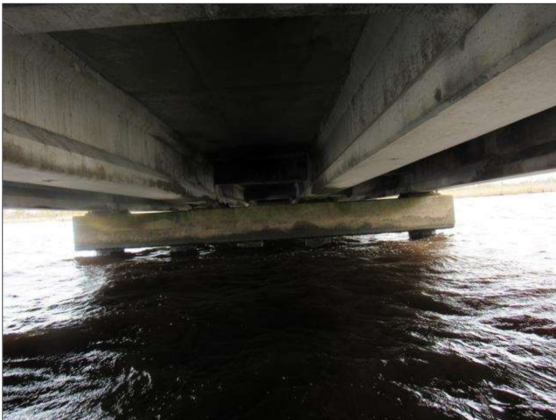
SUBSTRUCTURE TYPE 2, BENT 276 WEST FACE SHOWN
