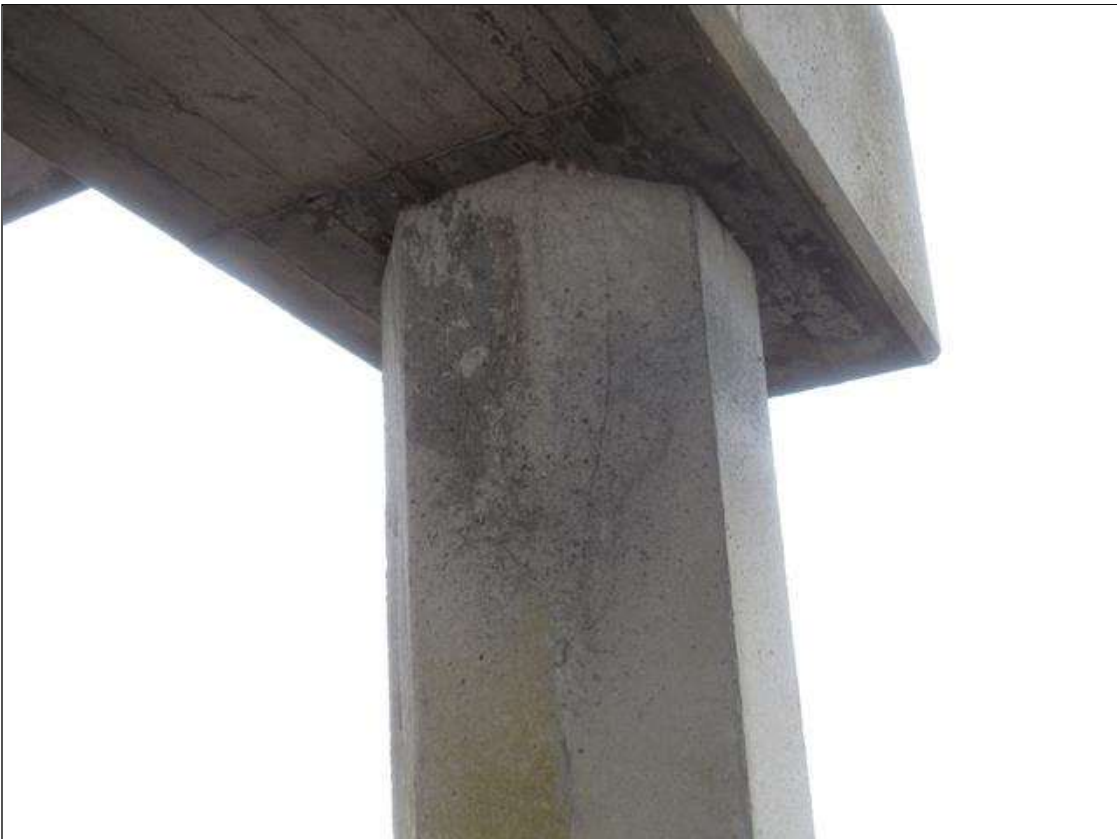
Bent 107 Pile 1: (PAR) (2) UP TO 2' X 0.025" VERTICAL CRACKS, SOUTH FACE, BEGINNING AT BOTTOM OF CAP WITH ADJACENT 2' X UP TO 1' DELAMINATION.
