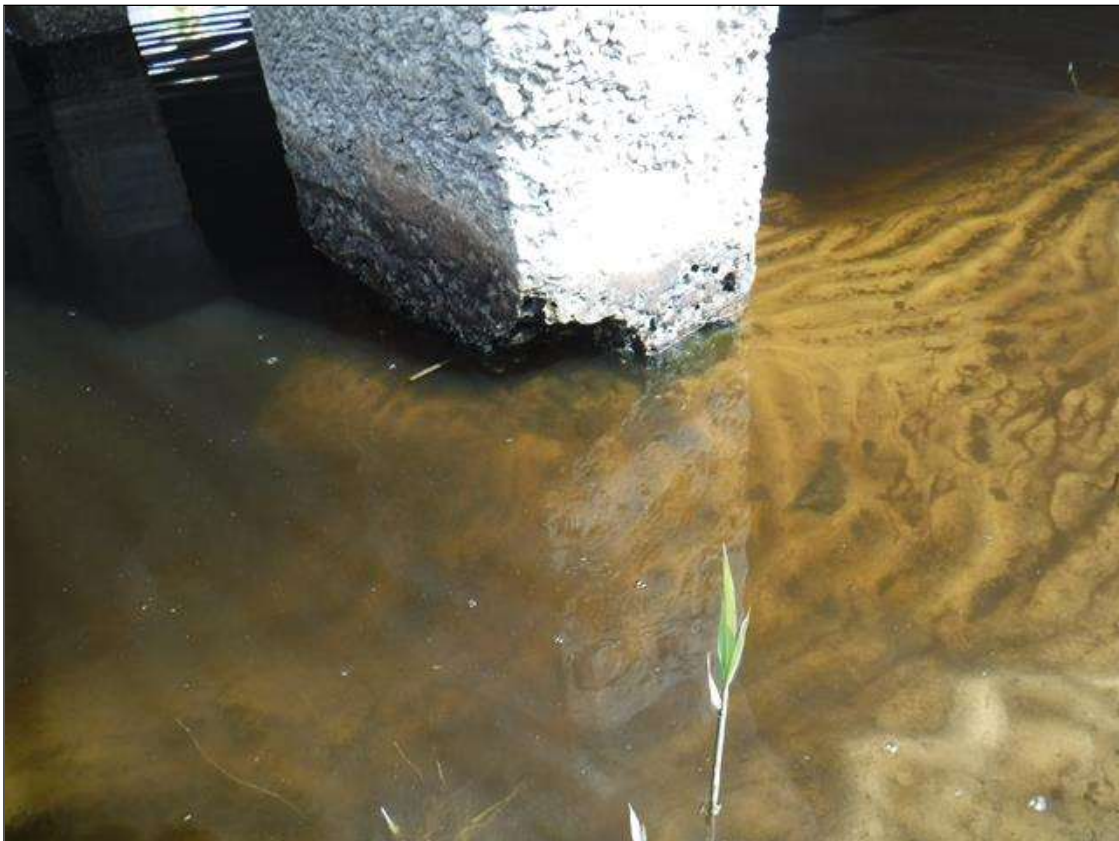
Bent 306 Pile 4: 8" X 8" X 8" SPALL AT BOTTOM SOUTH CORNER
