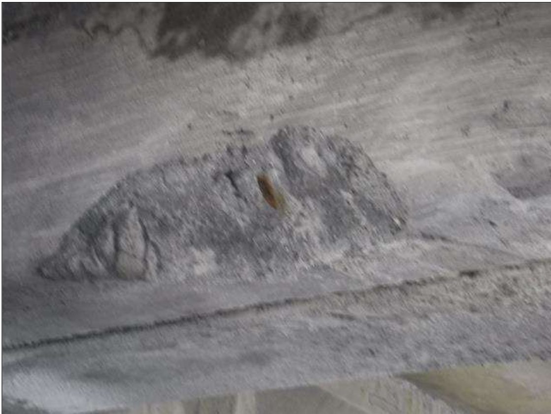
Span 181 Beam 3: 48" X 8" X 12" FAILED CORNER PATCHED AREA, WITH EXPOSED REINFORCING, END DIAPHRAGM, BETWEEN BEAMS 2 AND 3, EAST FACE, AT BENT 180.
