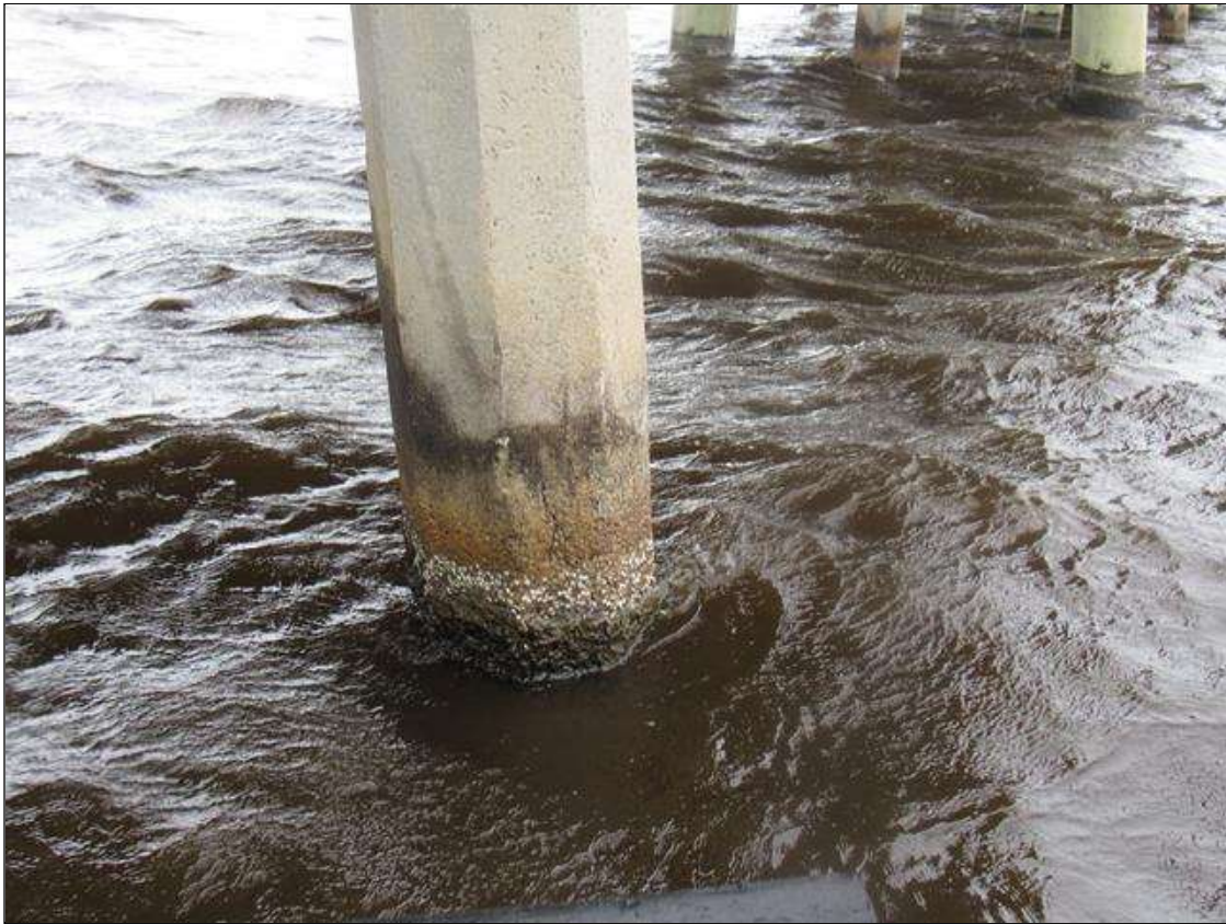
Bent 102 Pile 4: (PAR) UP TO 3' X 0.014" VERTICAL CRACKS, NORTH AND SOUTH FACES, BEGINNING 9' FROM BOTTOM OF CAP, WITH ADJACENT 3' X UP TO 2' DELAMINATION.
