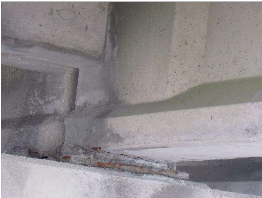
Span 33 Beam 2: 1' X 1' PATCHED AREA, SOUTH FACE, AT BENT 32.
