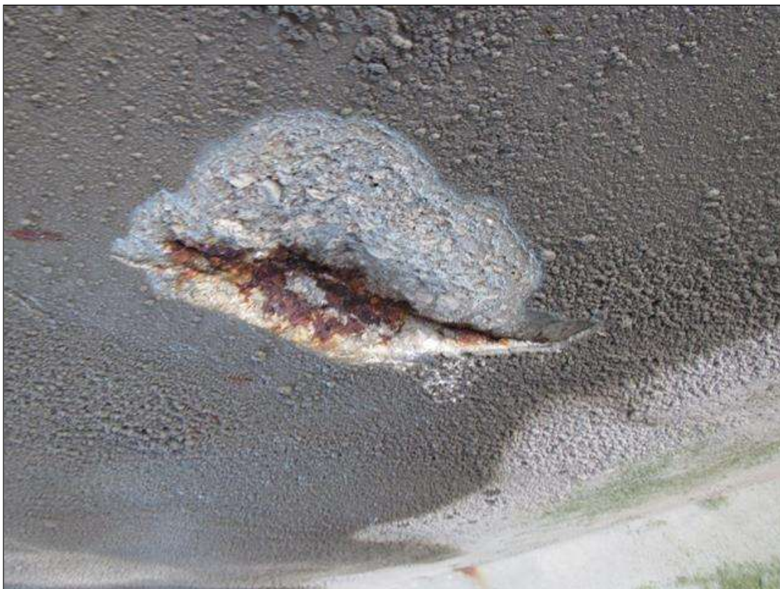
Span 285 Deck: (PAR) 12' DIAPHRAGM X 1/2" DEEP SPALL WITH EXPOSED REBAR ON BOTTOM FACE LOCATED NEAR MID-SPAN AND PILE 3
