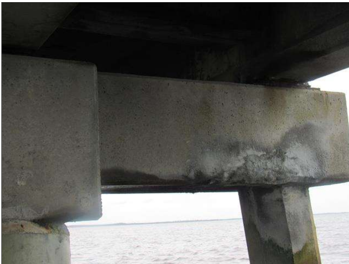
Bent 271 Cap 1: 4' X 6" PATCHED AREA, EAST FACE, BETWEEN BEAMS 1 AND 2.
