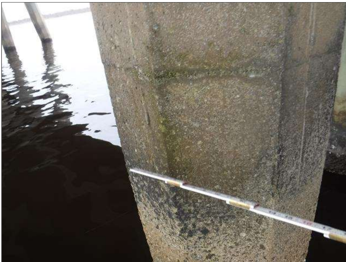
Bent 244 Pile 3: (PAR) HAIRLINE TO 1/16" CRACKS WITH SURROUNDING 36" X 8" DELAMINATION ON NORTH FACE, 8' BELOW CAP, DOWN 4', MULTIPLE FACES. SCALING TO 1" DEEP WITH LOOSE AGGREGATE FROM WATERLINE TO MUDLINE.
