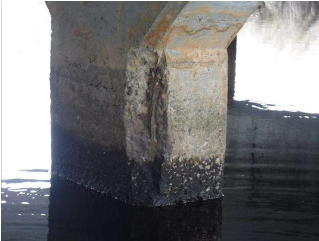
Bent 338 Pile 2: (PAR) 18" X 4" X UP TO 1" DEEP SPALL WITH EXPOSED REBAR, NORTHEAST CORNER. REBAR HAS 25% SECTION LOSS
