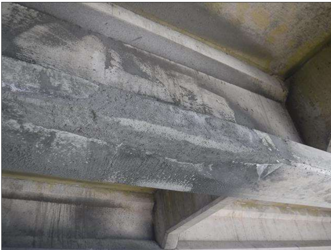
Span 20 Beam 3: 4' LONG X 12" TALL PATCHED AREA AT MIDPOINT OF SPAN.
