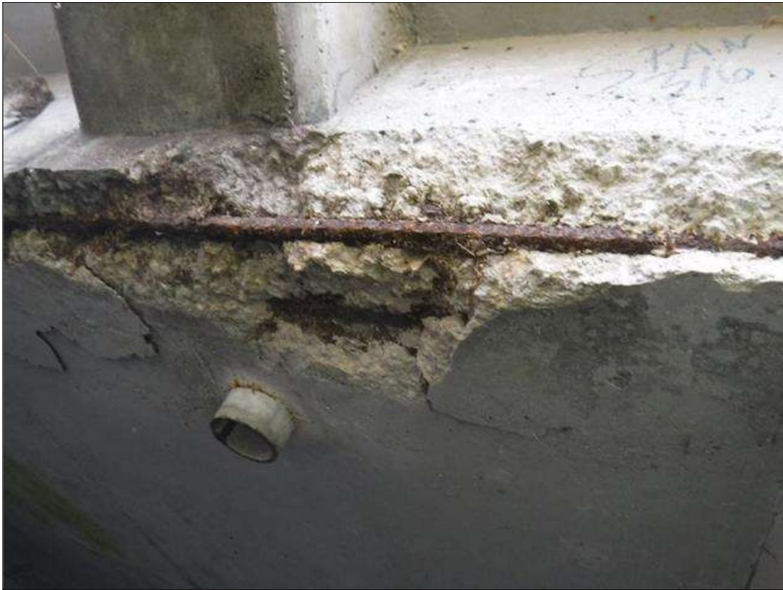
Span 316 Deck: (PAR) 40" X 12" X 6" DEEP SPALL WITH EXPOSED REBAR ON DECK UNDERSIDE, NORTH OVERHANG AT BENT 315
