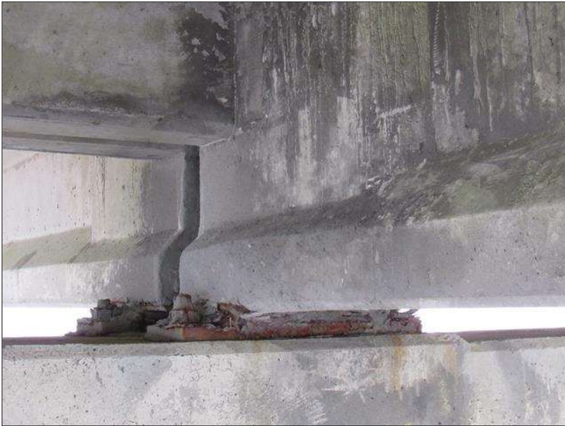
Span 58 Beam 3: 24" X 12" PATCHED AREA, NORTH FACE, AT BENT 58.
