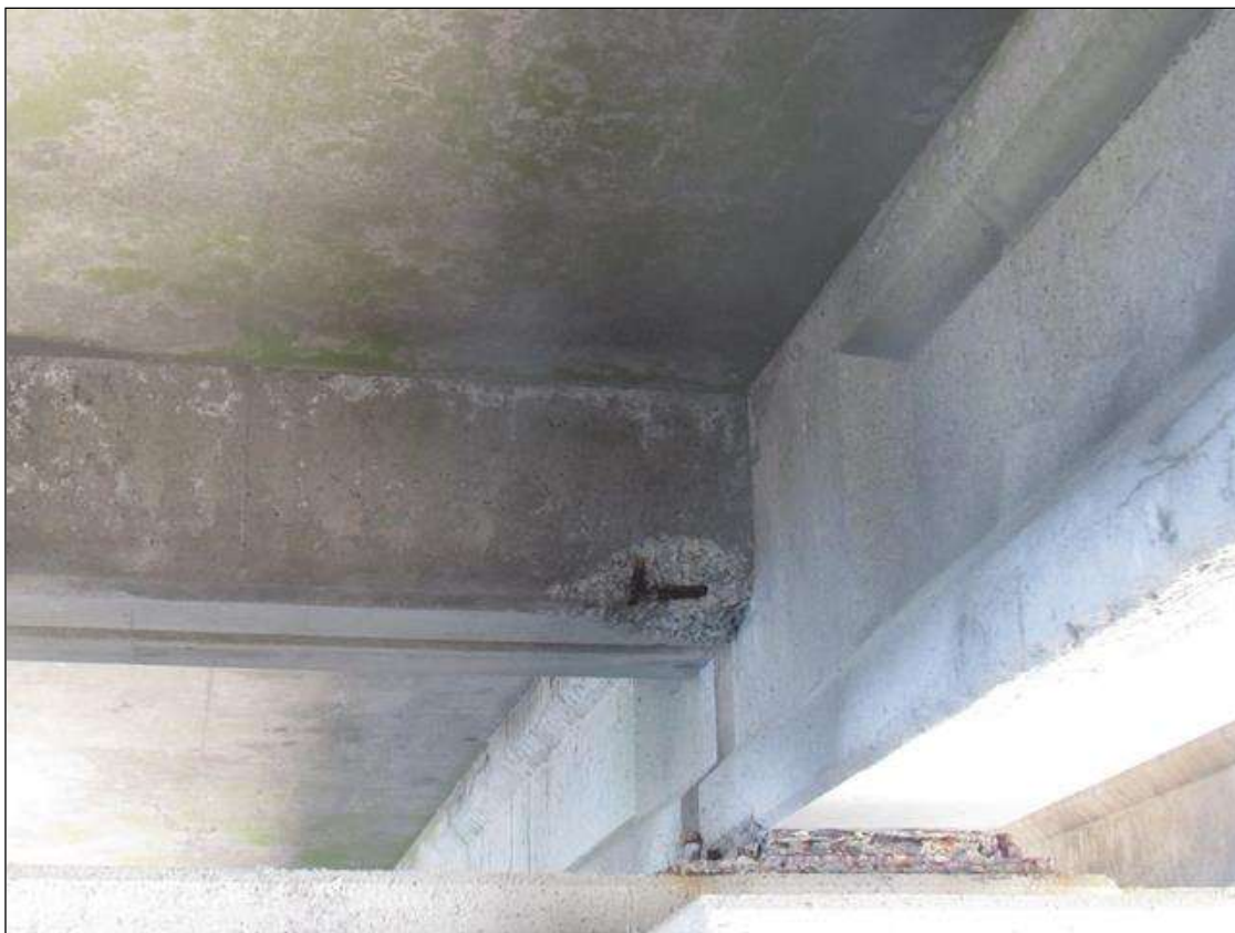
Span 5 Beam 3: 16" X 6" X 6" EDGE SPALL, WITH EXPOSED REINFORCING. WEST FACE OF BENT 5 DIAPHRAGM, BETWEEN BEAMS 2 AND 3.
