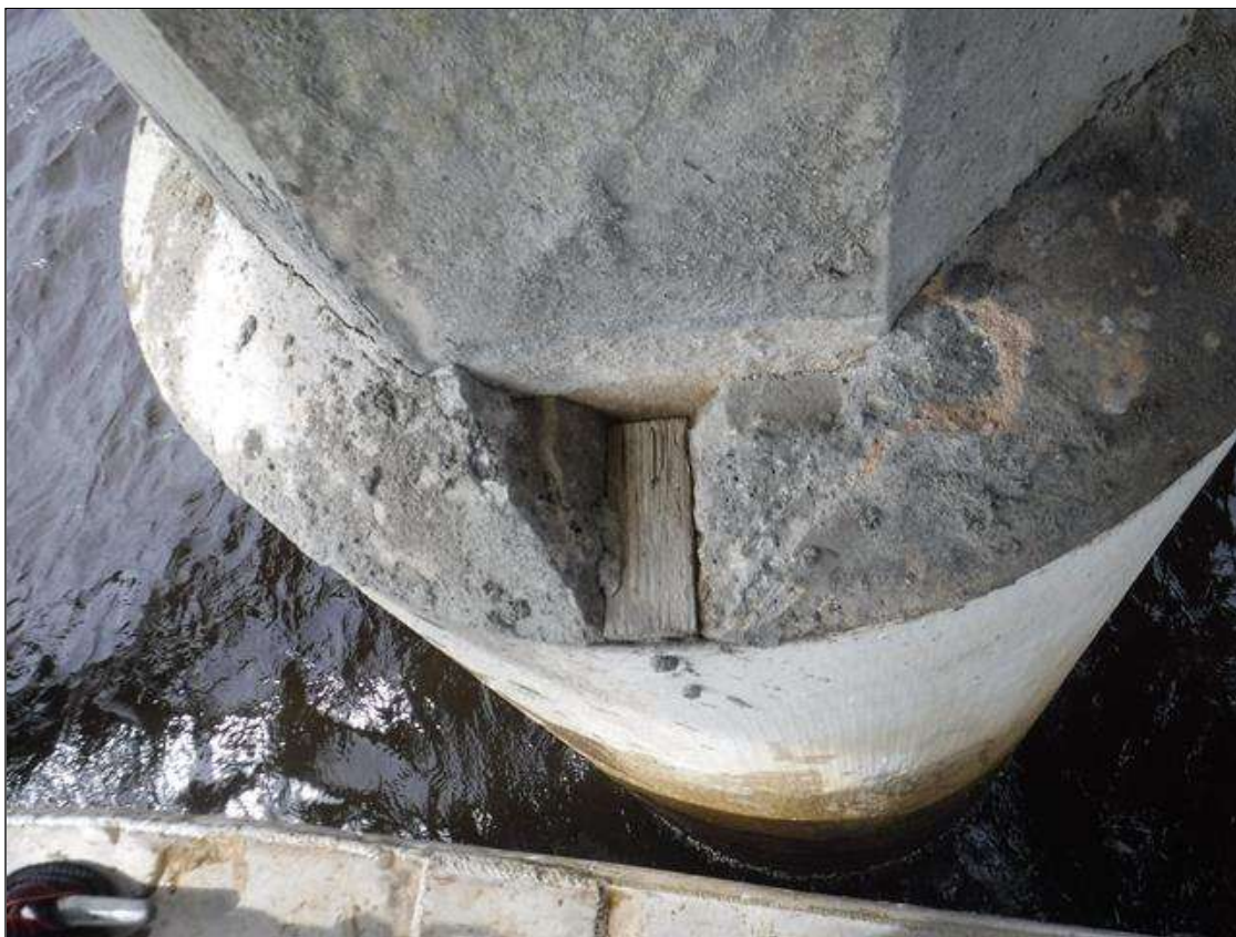
Bent 173 Pile 3: (2) UP TO 8" X 5" X 3" SPALLS, EAST AND WEST FACES, TOP OF PILE JACKET.
