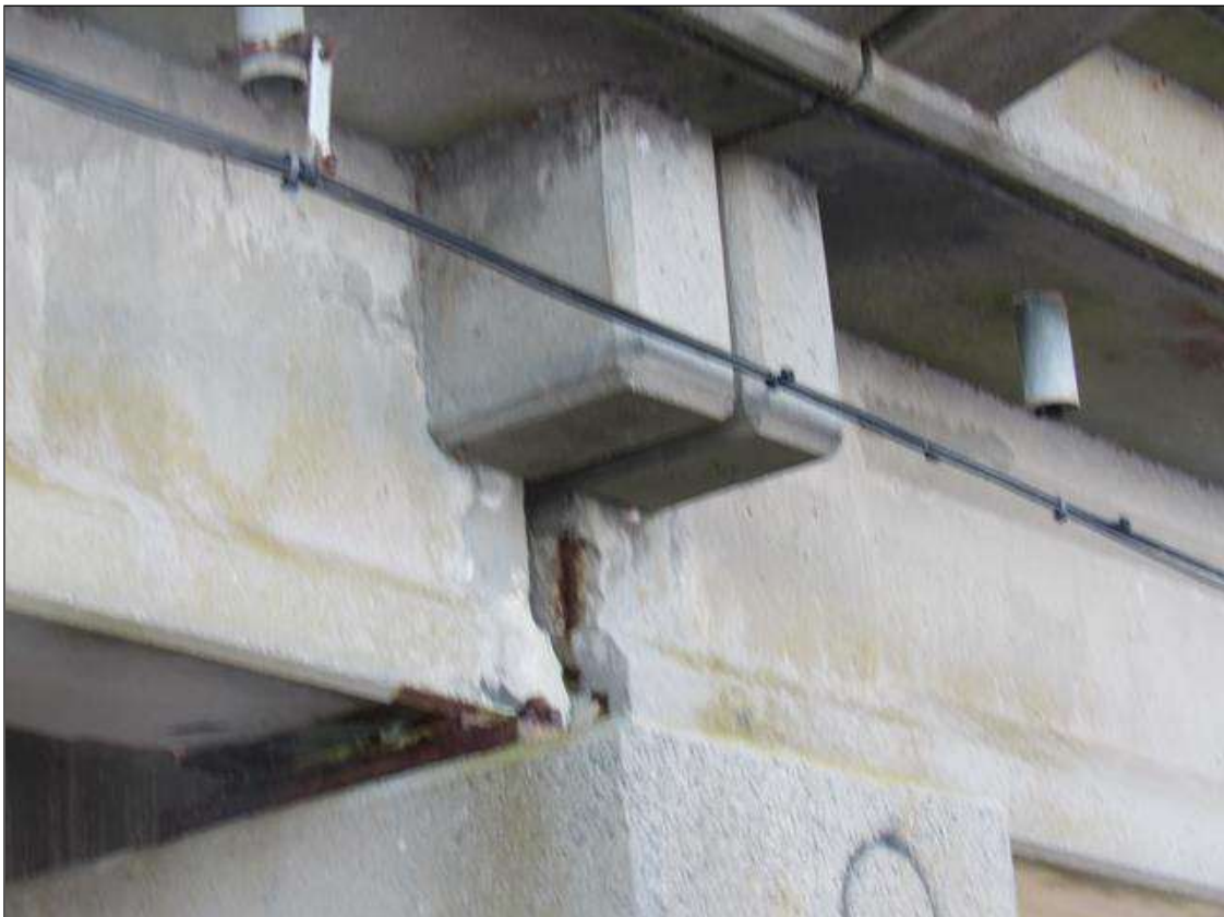
Span 8 Beam 1: 3" X 8" X 3" SPALL WITH EXPOSED REINFORCING, NORTH FACE, AT BENT 8.
