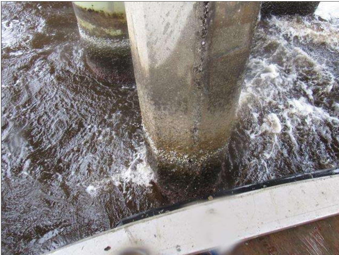
Bent 73 Pile 5: (PAR) (3) UP TO 3' X 0.25" VERTICAL CRACKS WITH SURROUNDING 3' X 1' DELAMINATION, BEGINNING 8' FROM BOTTOM OF CAP, AT RANDOM THROUGHOUT.
