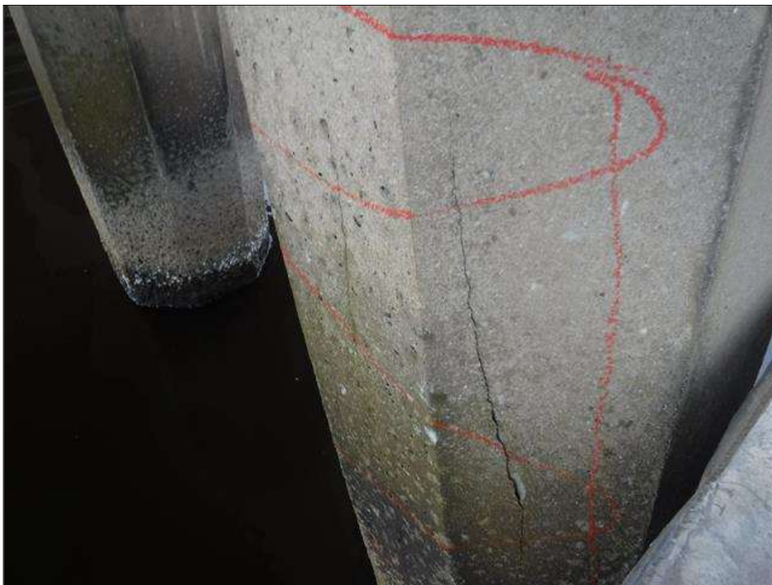
Bent 247 Pile 4: (PAR) HAIRLINE TO 1/8" CRACKS WITH 48" X 24" SURROUNDING DELAMINATION ON NORTH FACE, 8' BELOW CAP, DOWN 4' , MULTIPLE FACES. SCALING TO 1" DEEP WITH LOOSE AGGREGATE FROM WATERLINE TO MUDLINE.
