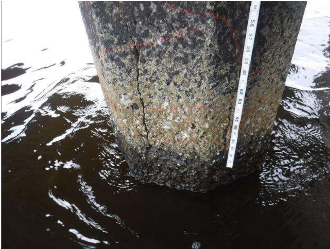
Bent 226 Pile 2: (PAR) HAIRLINE TO 1/8" CRACKS WITH ADJACENT 2' X 2' DELAMINATION, 8' BELOW CAP, DOWN 4', MULTIPLE FACES. SCALING TO 1" DEEP WITH LOOSE AGGREGATE FROM WATERLINE TO MUDLINE.
