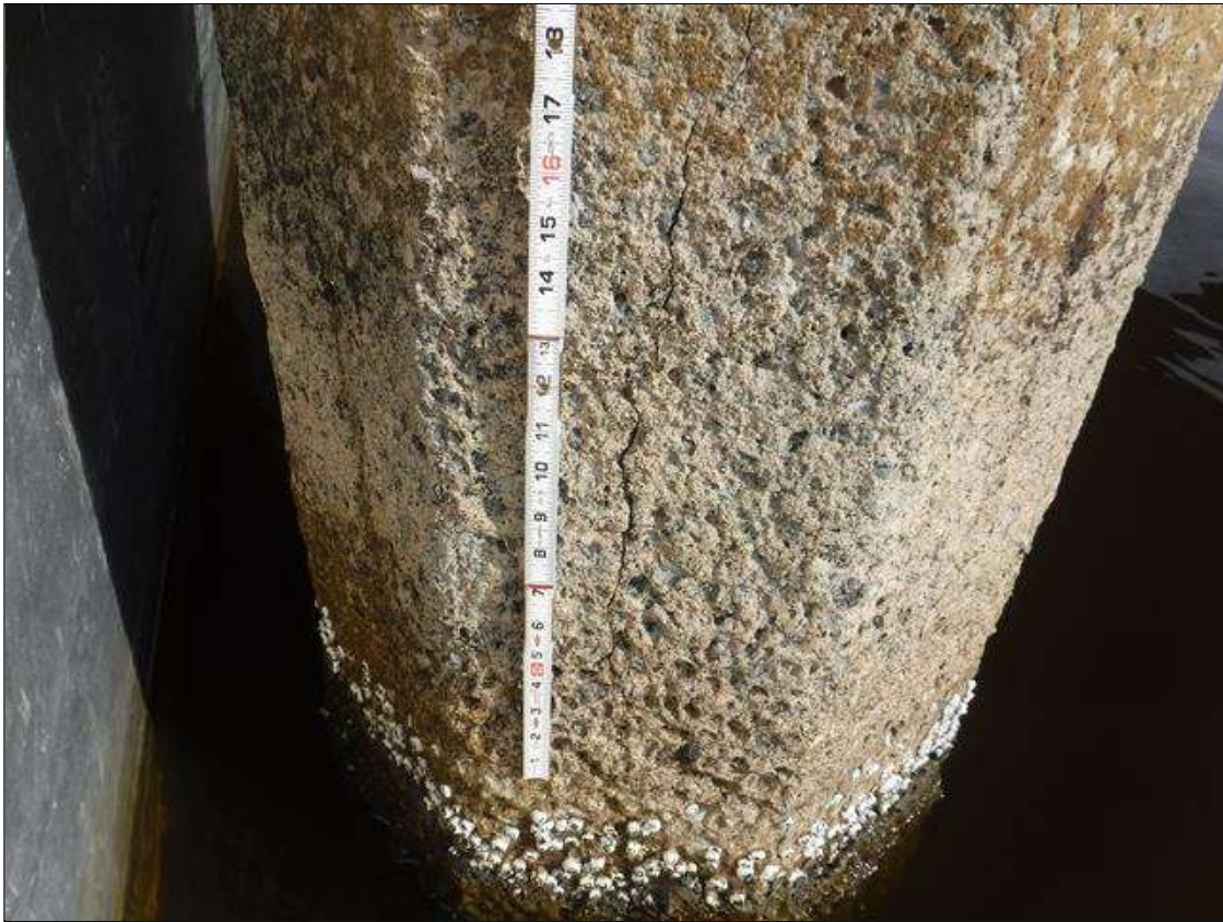
Bent 215 Pile 6: (PAR) (3) UP TO 2' X 0.025" VERTICAL CRACKS, SOME WITH RUST STAINING, NORTH FACE, STARTING 8' FROM BOTTOM OF CAP.
