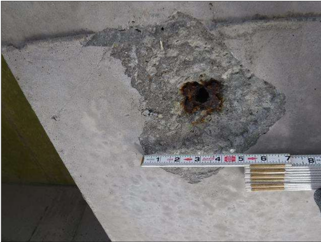
Span 217 Beam 3: 1' DIAMETER X 1/2" DEEP SPALL ON BOTTOM FACE AT MIDPOINT OF SPAN.
