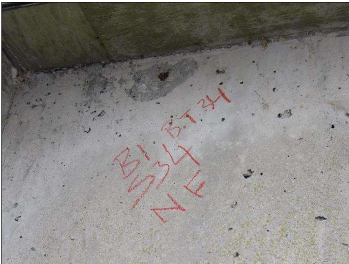
Span 34 Beam 1: 5" DIAMETER X 1/2" DEEP DELAMINATION WITH EXPOSED REBAR ON NORTH FACE OF WEB AT BENT 34
