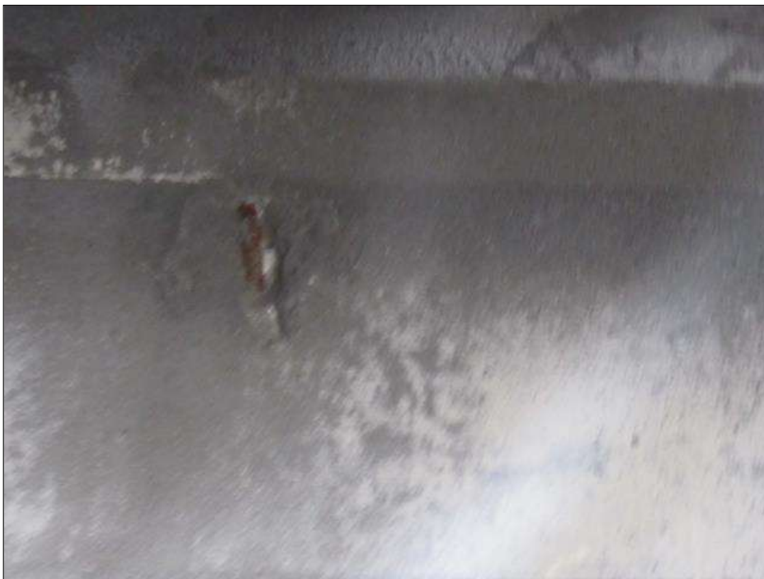
Span 1 Beam 2: 8" X 8" X 1" SPALL, WITH EXPOSED REINFORCING, SOUTH FACE, 16" FROM END BENT 1.
