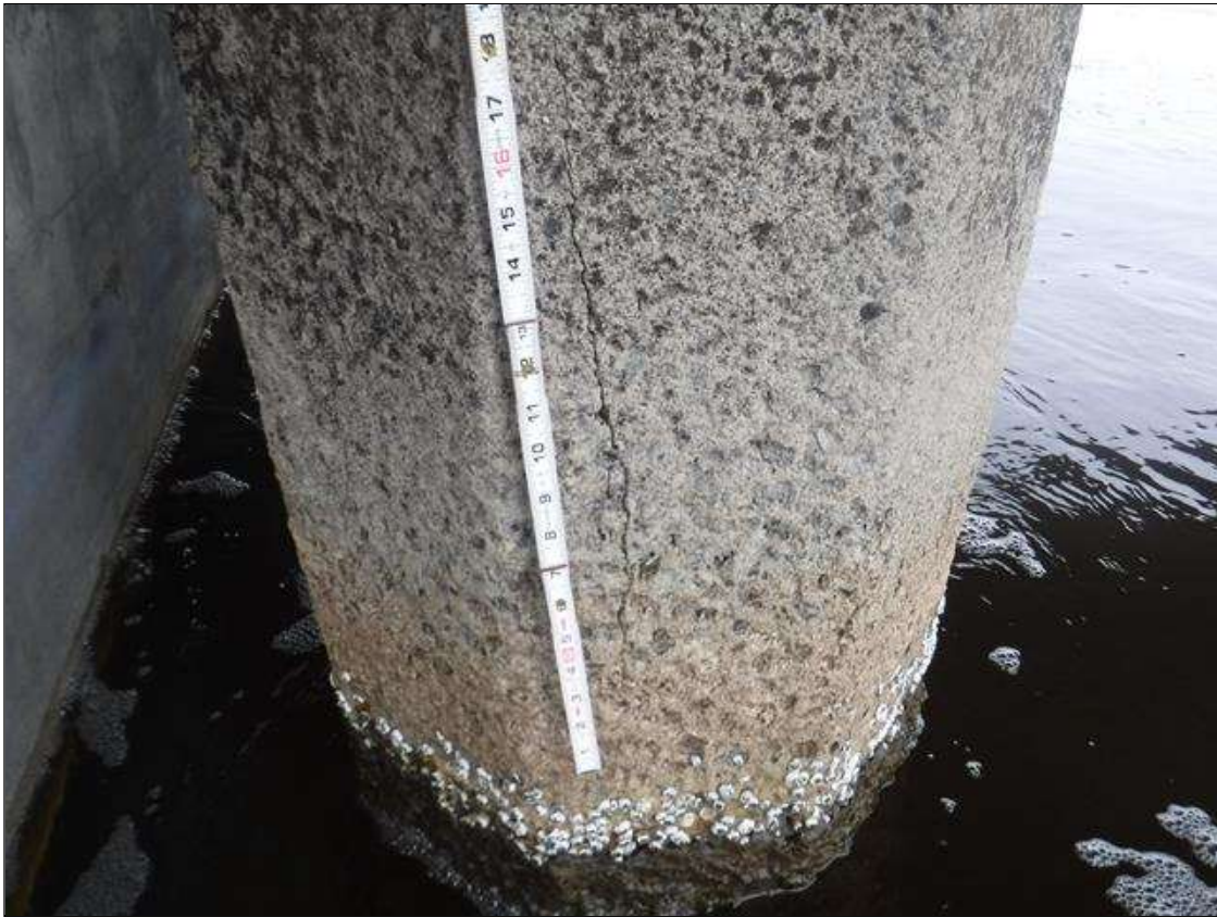
Bent 236 Pile 5: (PAR) (3) UP TO 3' X 0.06" VERTICAL CRACKS, BEGINNING 7' FROM BOTTOM OF CAP, AT RANDOM THROUGHOUT.
