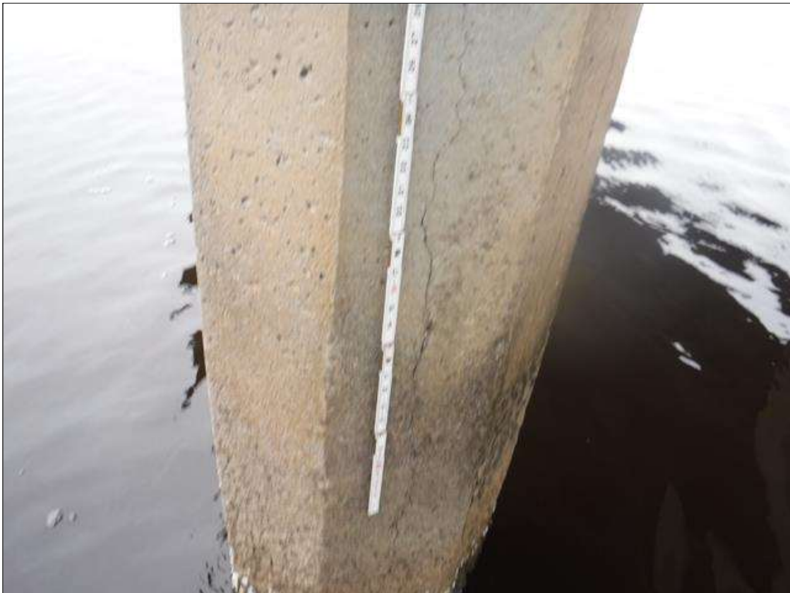
Bent 243 Pile 6: (PAR) (2) UP TO 10' X 0.03" VERTICAL CRACKS, EAST FACE, BEGINNING AT BOTTOM OF CAP.
