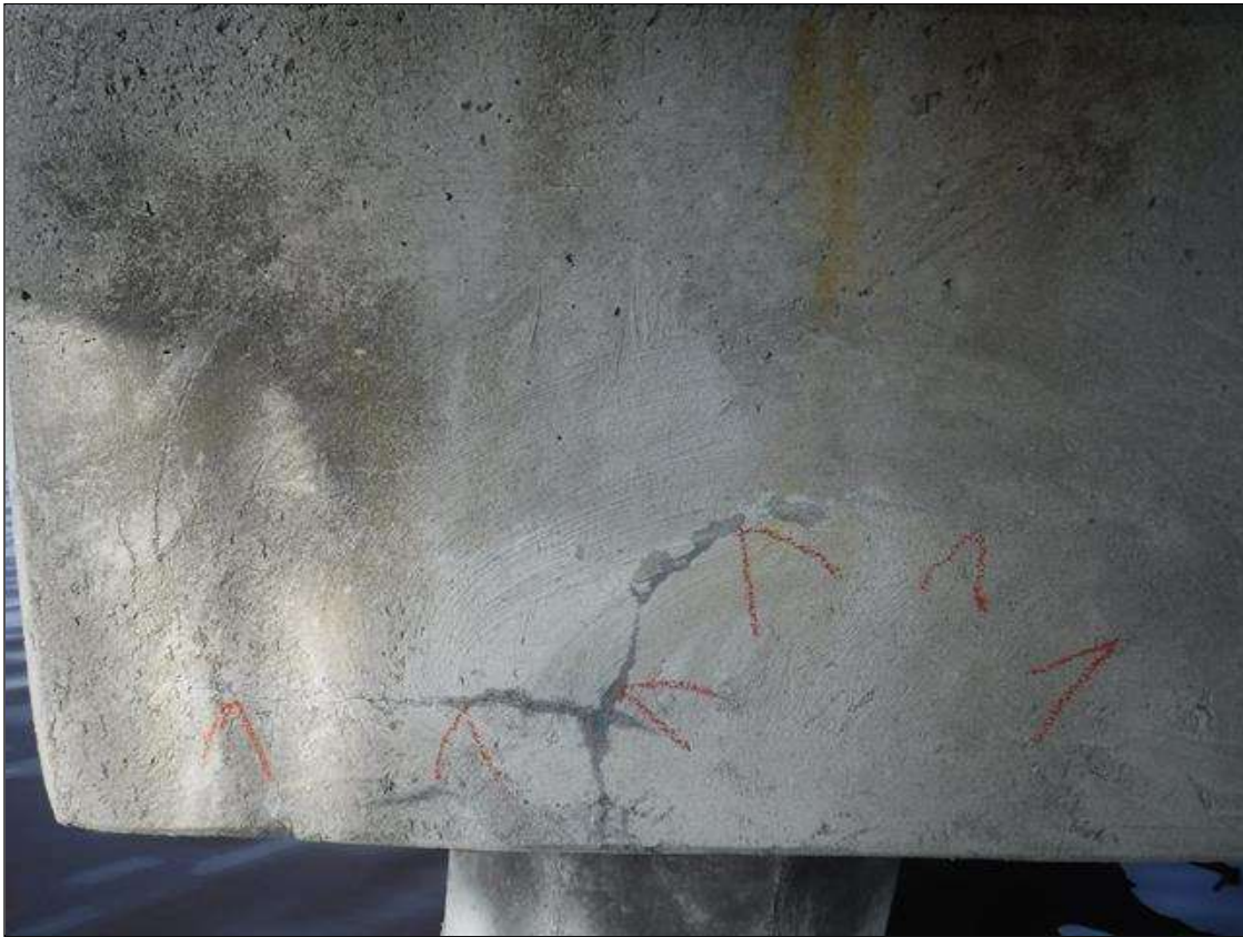
Bent 78 Cap 1: 3' HAIRLINE CRACK ON EAST FACE OVER PILE 4
