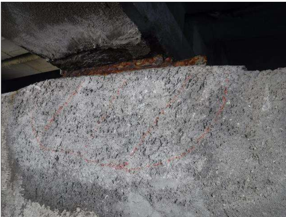
Bent 10 Cap 1: 2' X 1' FAILED PATCHED AREA BELOW BEAM 2
