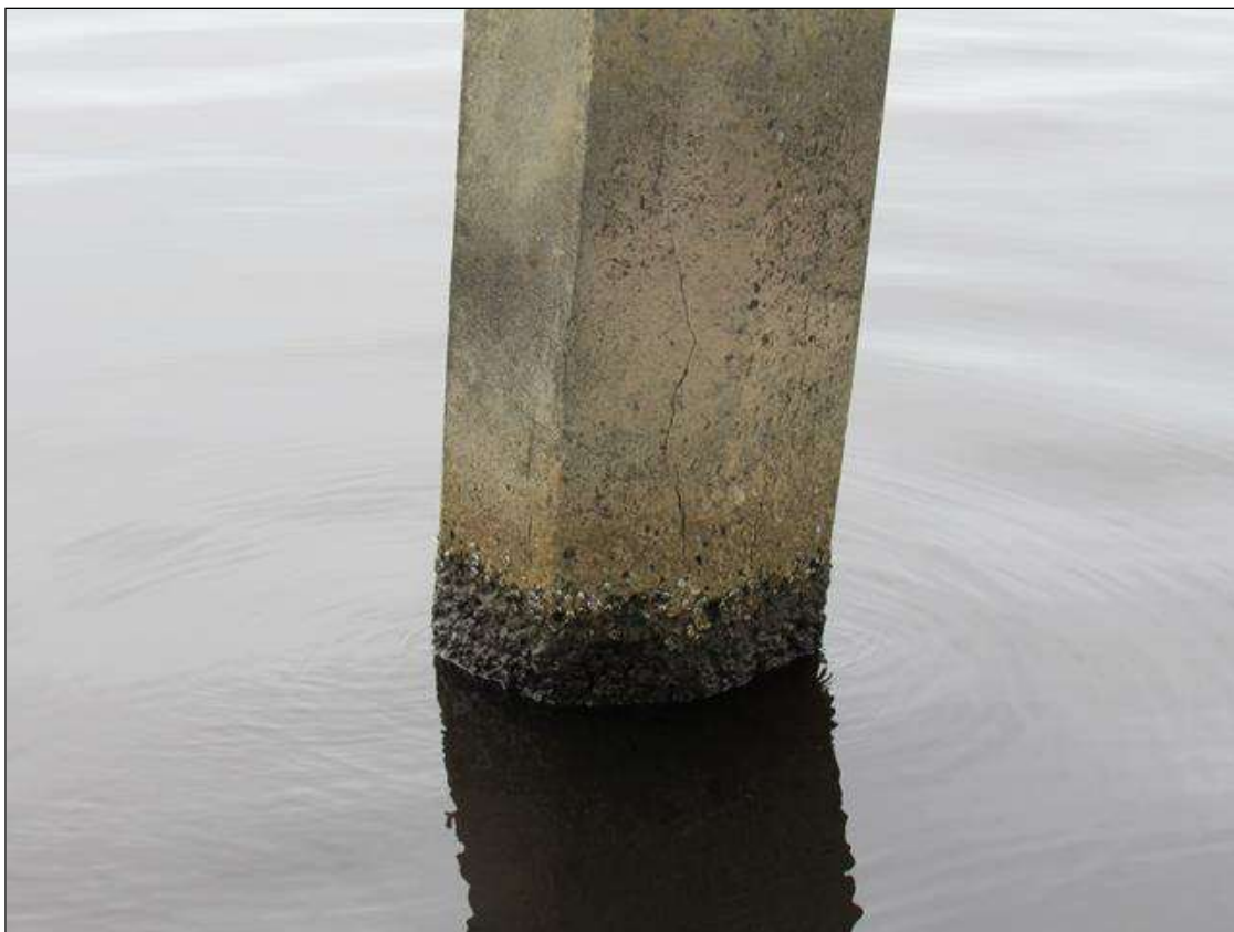
Bent 31 Saved Pile 1: 2' X 1' DELAMINATION, SOUTH FACE, 8' FROM BOTTOM OF CAP.
