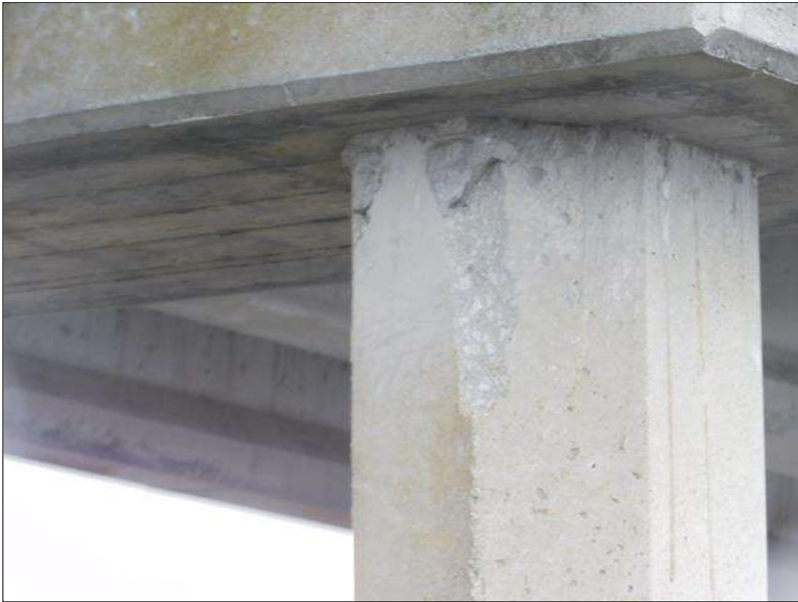
Bent 95 Saved Pile 4: 16" X 4" X 3/4" SPALL, WEST FACE, AT BOTTOM OF CAP.
