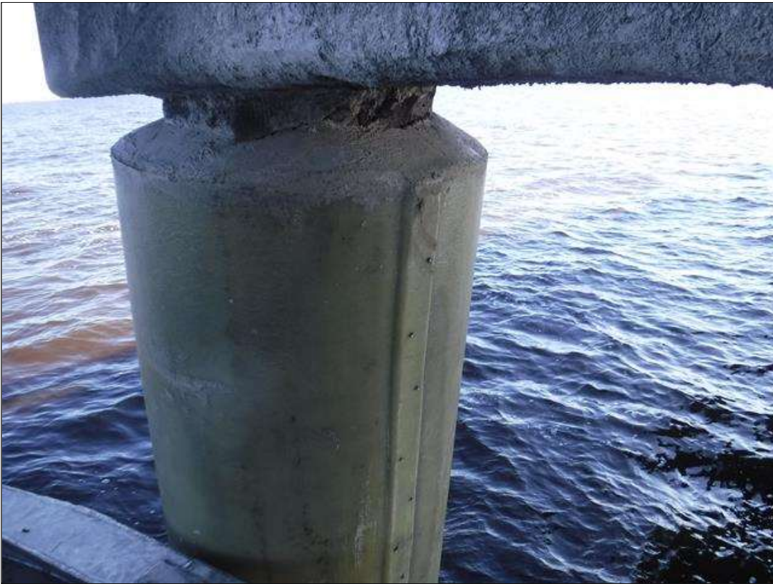
Bent 11 Saved Pile 1: PILE REPAIRED WITH 3' DIAMETER CONCRETE JACKET STARTING 6" BELOW BOTTOM OF CAP
