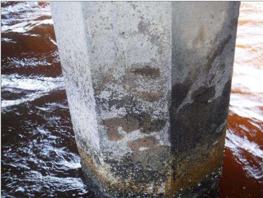
Bent 25 Saved Pile 3: (PAR) HAIRLINE TO 1/8" CRACK, 8' BELOW CAP, DOWN 5', EAST QUAD. SCALING TO 1" DEEP FROM WATERLINE TO MUDLINE.
