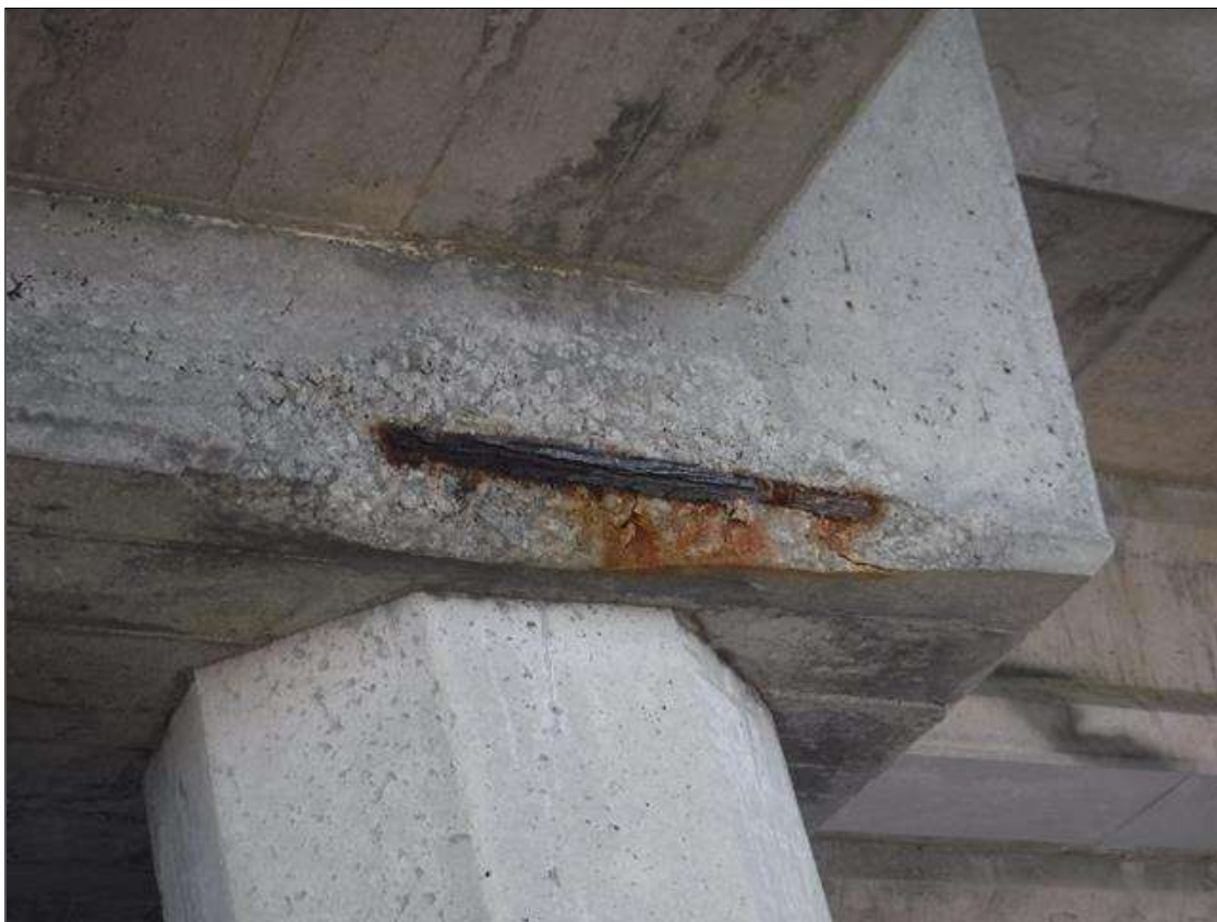
Bent 29 Cap 1: (PAR) 4" LONG, 16" WIDE, AND 3" DEEP SPALL WITH EXPOSED REBAR ON NORTH FCE ABOVE PILE 5. REBAR HAS 15% SECTION LOSS
