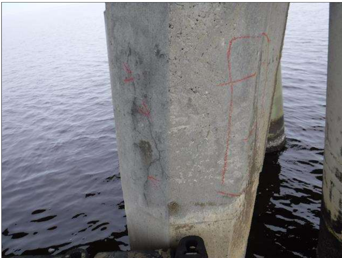
Bent 231 Pile 4: UP TO 3' CRACKED PATCHED AREA WITH 2' X 8" DELAMINATION AROUND THE PILE, WITH RUST STAINING, 5' FROM BOTTOM OF CAP.
