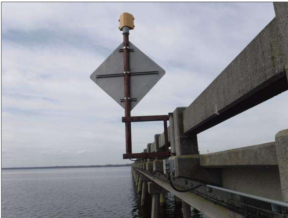
UTILITY AND SIGN CONNECTION TO SOUTH OVERHANG AT BENT 99
