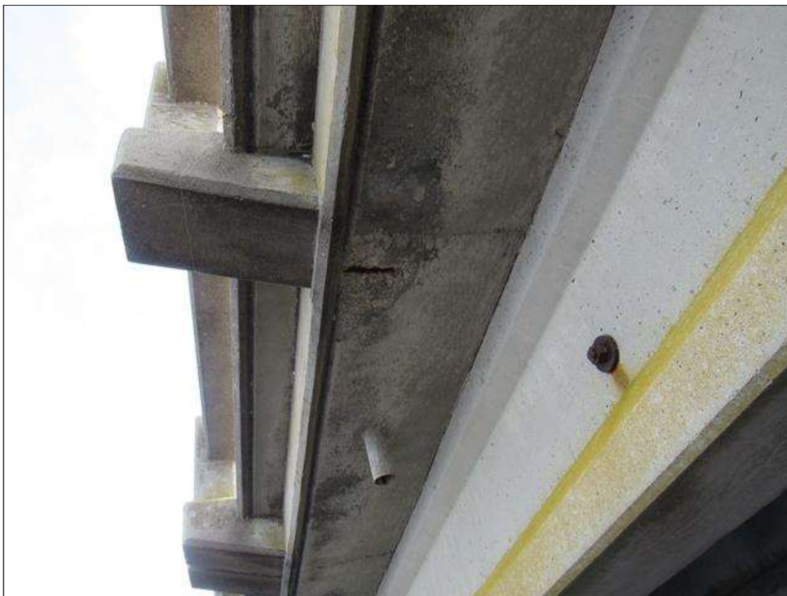
Span 276 Deck: 18" X 10" X 1" SPALL WITH EXPOSED REINFORCING, DECK UNDERSIDE, NORTH OVERHANG, NEAR MIDSPAN.
