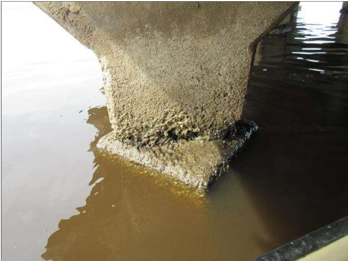
Bent 287 Pile 4: (PAR) 6" X 12" X 20" SPALL, WITH EXPOSED PRIMARY REBAR, NORTH FACE, 2' FROM BOTTOM OF CAP.
