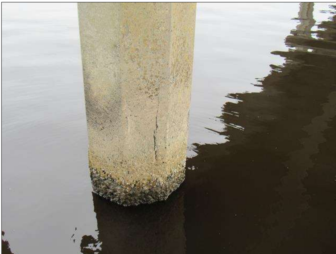
Bent 31 Saved Pile 2: (PAR) UP TO 1/4" VERTICAL CRACK, 8' BELOW CAP, DOWN 6', SOUTH FACE. SCALING TC 1" DEEP FROM WATERLINE TO MUDLINE.
