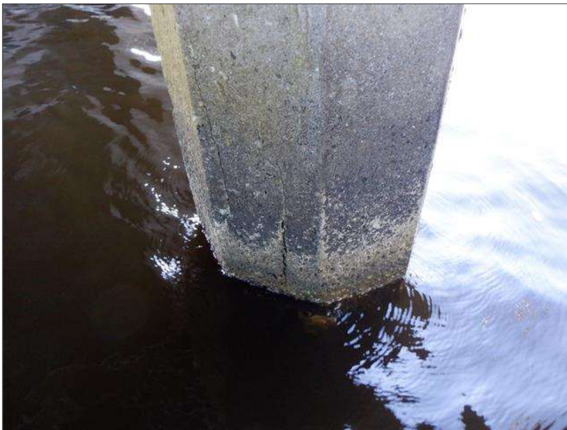
Bent 271 Pile 6: UW (PAR): H/L TO 1/8" CRACKS MULTIPLE FACES, FROM ABOVE THE HIGH WATER MARK DOWN THROUGH THE SPASH ZONE AND TAPERING TO HAIRLINE 1' TO 3' BELOW THE WATERLINE. SCALING TO 1" DEEP FROM WATERLINE TO MUDLINE.
