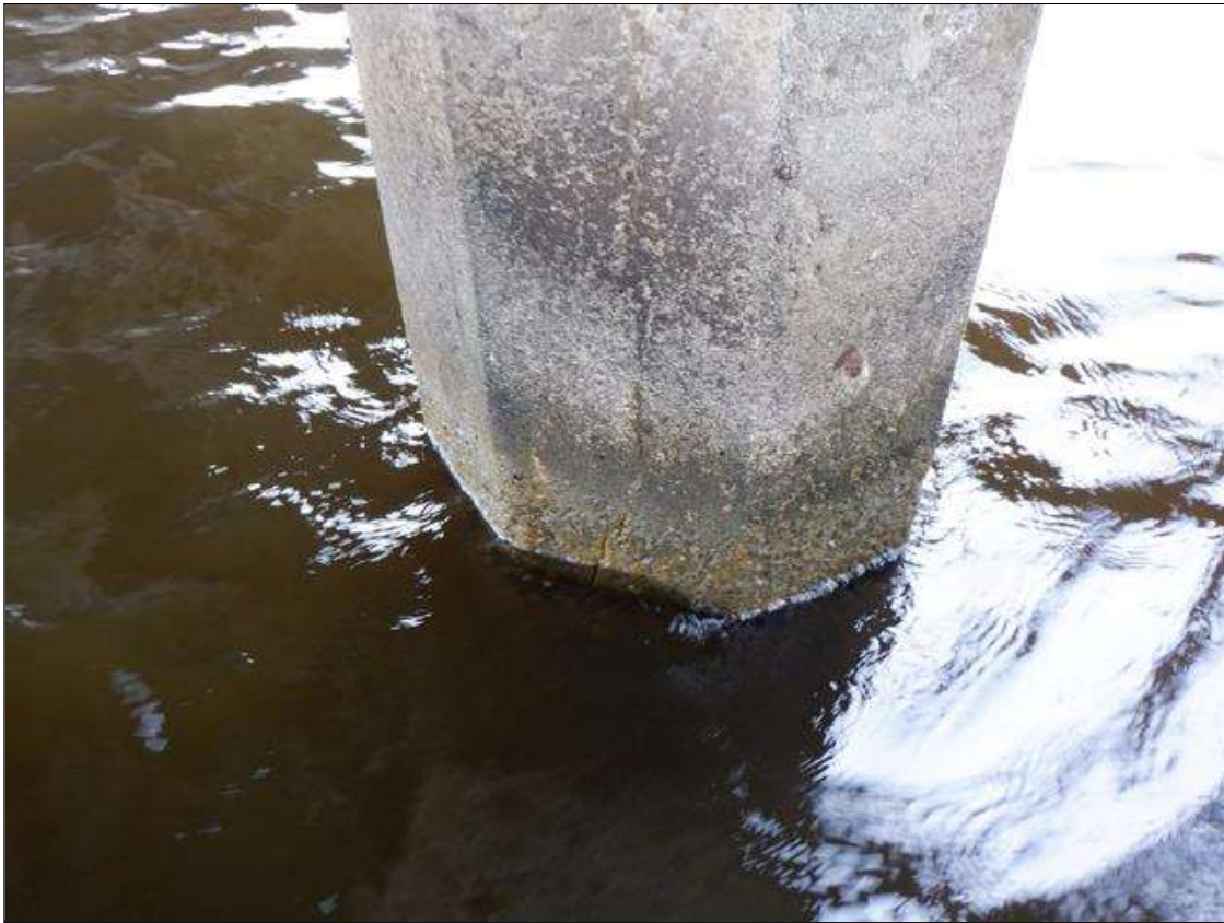
Bent 31 Saved Pile 3: UW (PAR): H/L TO 1/8" CRACKS MULTIPLE FACES, FROM ABOVE THE HIGH WATER MARK DOWN THROUGH THE SPASH ZONE AND TAPERING TO HAIRLINE 1' TO 3' BELOW THE WATERLINE. SCALING TO 1" DEEP FROM WATERLINE TO MUDLINE.
