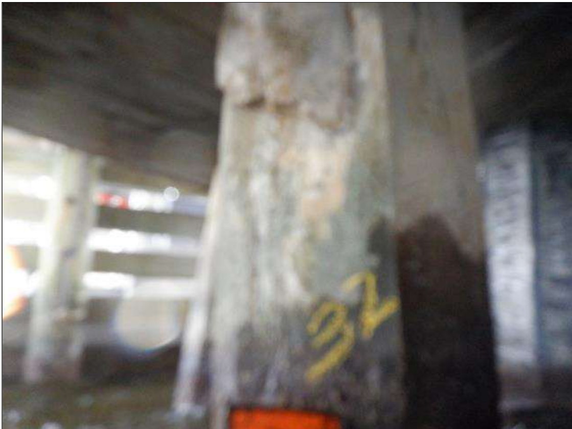
Bent 116 PIVOT Pile 32: U/W (PAR): CRACKED TO 1/8", DELAMINATED 1" TO 3" DEEP, MULTIPLE FACES, FROM CAP DOWN 4'. SCALING TO 1" DEEP FROM WATERLINE TO MUDLINE.
