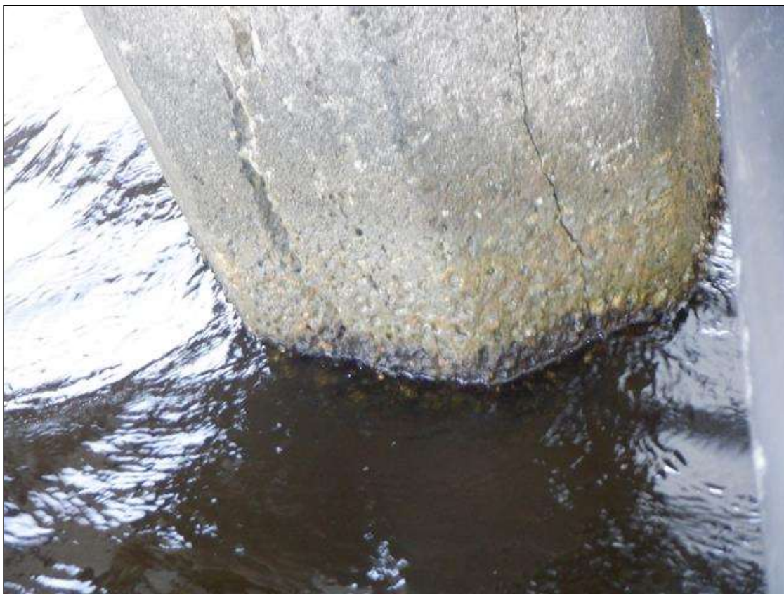
Bent 41 Saved Pile 2: UW (PAR): H/L TO 1/8" CRACKS MULTIPLE FACES, FROM ABOVE THE HIGH WATER MARK DOWN THROUGH THE SPASH ZONE AND TAPERING TO HAIRLINE 1' TO 3' BELOW THE WATERLINE. SCALING TO 1" DEEP FROM WATERLINE TO MUDLINE.
