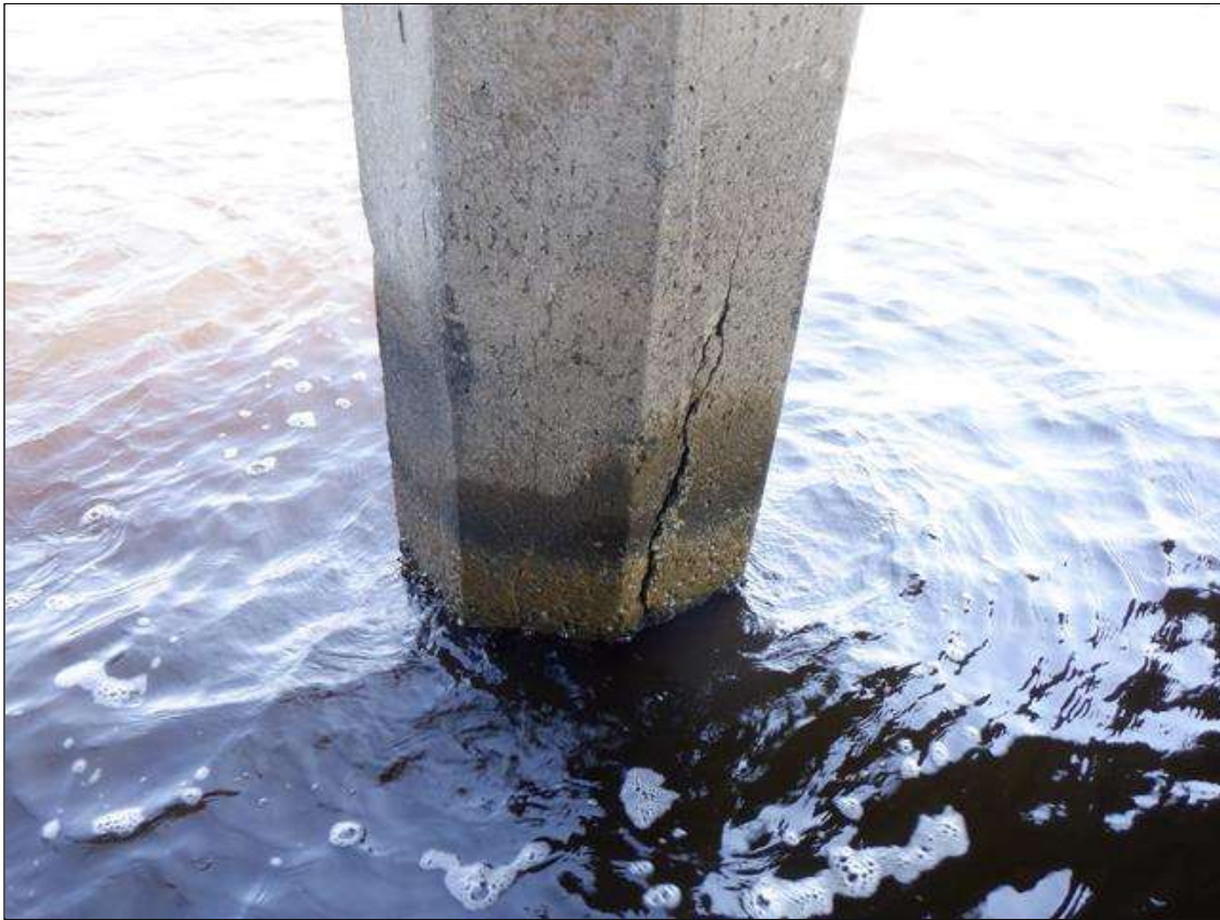
Bent 46 Saved Pile 4: UW (PAR): H/L TO 1/8" CRACKS MULTIPLE FACES, FROM ABOVE THE HIGH WATER MARK DOWN THROUGH THE SPASH ZONE AND TAPERING TO HAIRLINE 1' TO 3' BELOW THE WATERLINE. SCALING TO 1" DEEP FROM WATERLINE TO MUDLINE.
