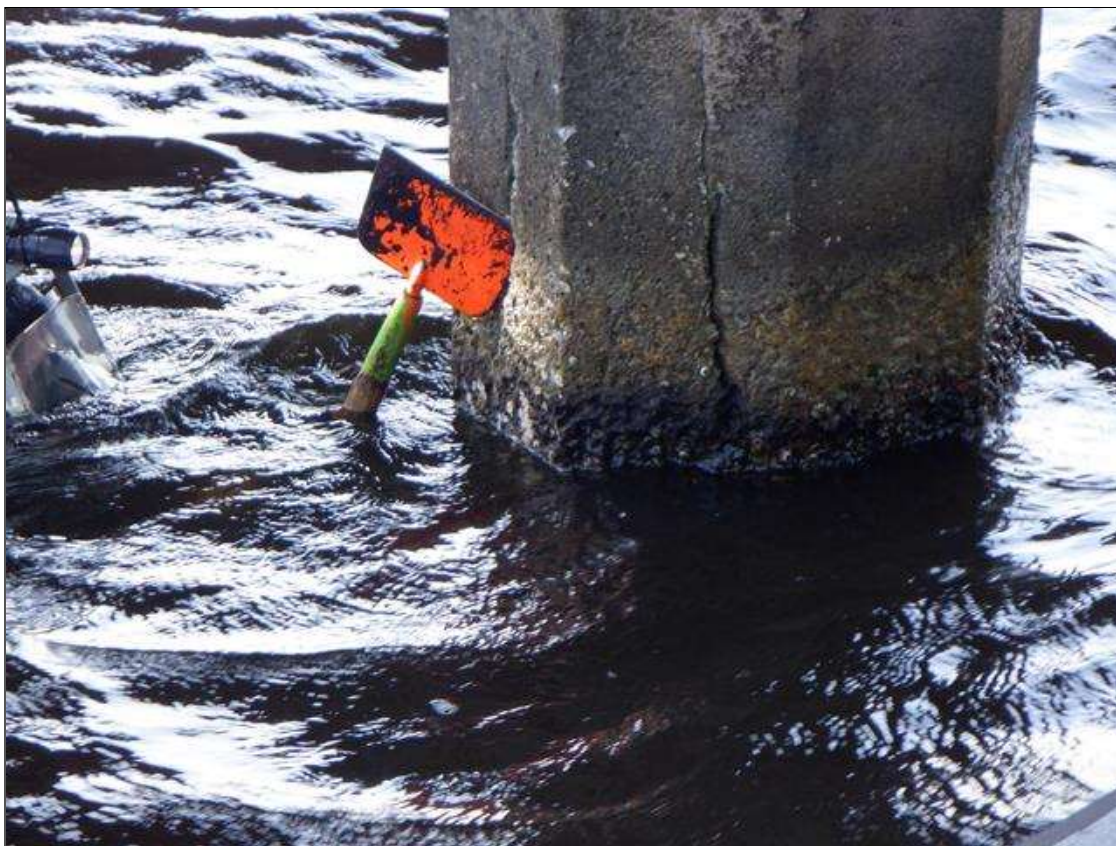
Bent 49 Saved Pile 3: UW (PAR): H/L TO 1/8" CRACKS MULTIPLE FACES, FROM ABOVE THE HIGH WATER MARK DOWN THROUGH THE SPASH ZONE AND TAPERING TO HAIRLINE 1' TO 3' BELOW THE WATERLINE. SCALING TO 1" DEEP FROM WATERLINE TO MUDLINE.
