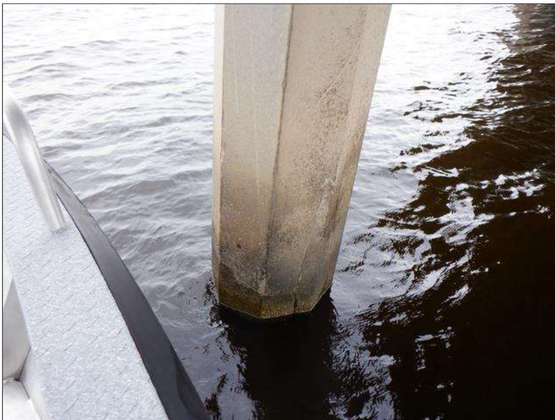
Bent 47 Saved Pile 4: UW (PAR): H/L TO 1/8" CRACKS MULTIPLE FACES, FROM ABOVE THE HIGH WATER MARK DOWN THROUGH THE SPASH ZONE AND TAPERING TO HAIRLINE 1' TO 3' BELOW THE WATERLINE. SCALING TO 1" DEEP FROM WATERLINE TO MUDLINE.
