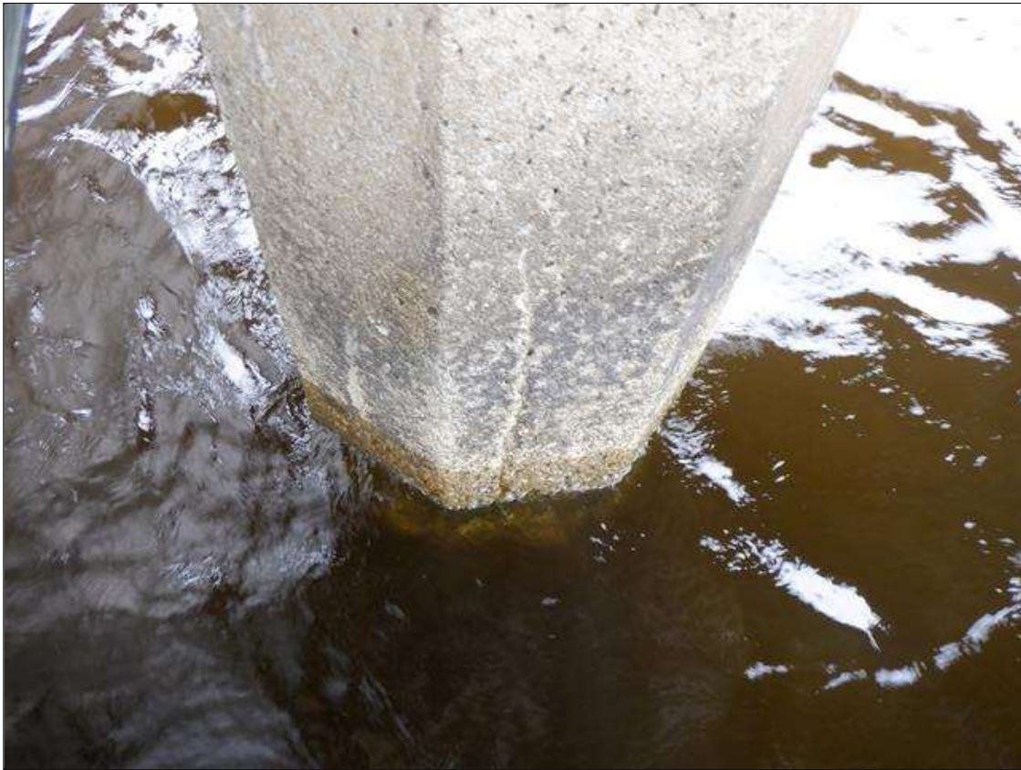
Bent 194 Pile 3: UW (PAR): H/L TO 1/8" CRACKS MULTIPLE FACES, FROM ABOVE THE HIGH WATER MARK DOWN THROUGH THE SPASH ZONE AND TAPERING TO HAIRLINE 1' TO 3' BELOW THE WATERLINE. SCALING TO 1" DEEP FROM WATERLINE TO MUDLINE.
