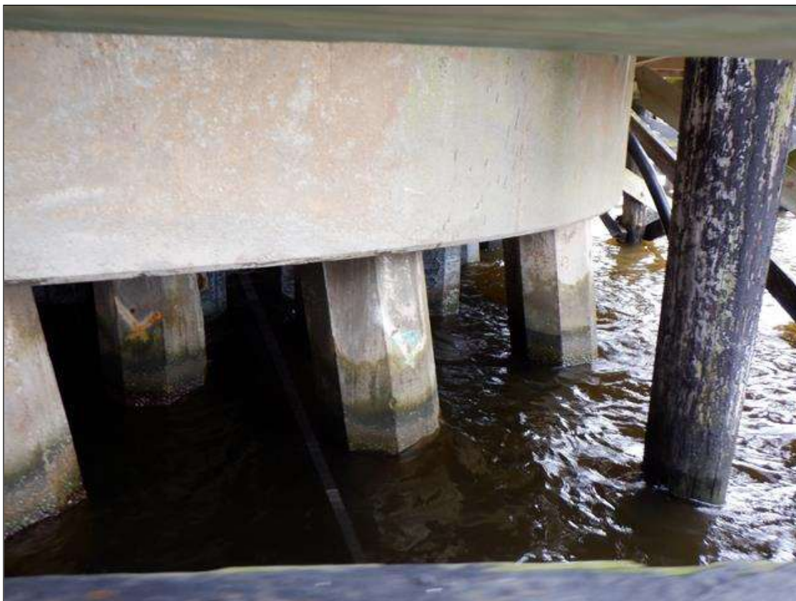
PIVOT BENT AND PILES
