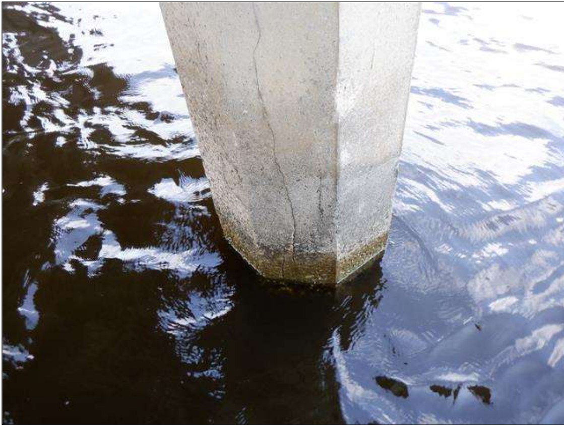
Bent 31 Saved Pile 1: UW (PAR): H/L TO 1/8" CRACKS MULTIPLE FACES, FROM ABOVE THE HIGH WATER MARK DOWN THROUGH THE SPASH ZONE AND TAPERING TO HAIRLINE 1' TO 3' BELOW THE WATERLINE. SCALING TO 1" DEEP FROM WATERLINE TO MUDLINE.
