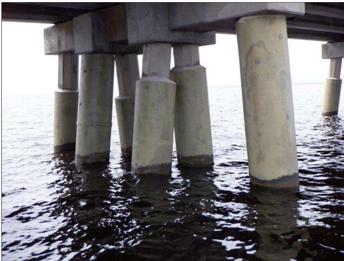
6-PILE BATTERED BENT
