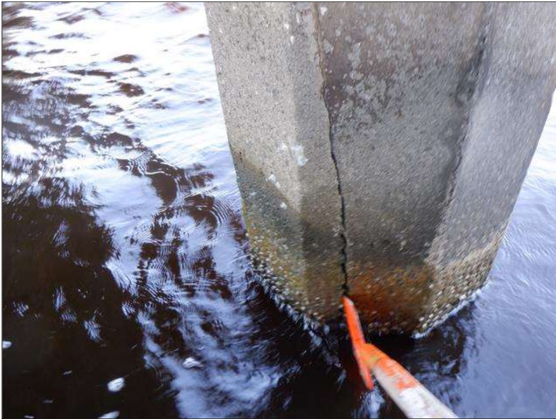
Bent 35 Saved Pile 1: UW (PAR): H/L TO 1/8" CRACKS MULTIPLE FACES, FROM ABOVE THE HIGH WATER MARK DOWN THROUGH THE SPASH ZONE AND TAPERING TO HAIRLINE 1' TO 3' BELOW THE WATERLINE. SCALING TO 1" DEEP FROM WATERLINE TO MUDLINE.
