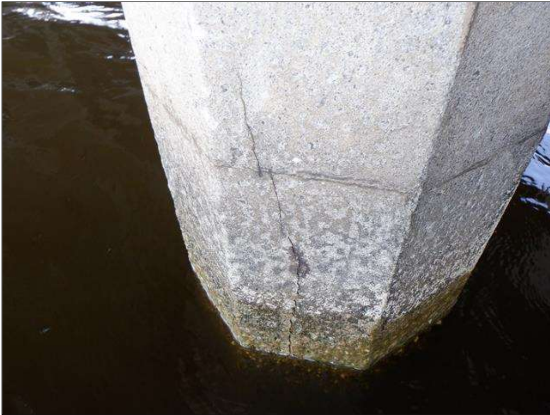
Bent 28 Saved Pile 3: UW (PAR): H/L TO 1/8" CRACKS MULTIPLE FACES, FROM ABOVE THE HIGH WATER MARK DOWN THROUGH THE SPASH ZONE AND TAPERING TO HAIRLINE 1' TO 3' BELOW THE WATERLINE. SCALING TO 1" DEEP FROM WATERLINE TO MUDLINE.
