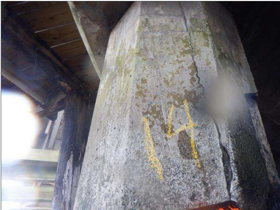
Bent 116 PIVOT Pile 14: U/W (PAR): CRACKED TO 1/8", DELAMINATED 1" TO 3" DEEP, MULTIPLE FACES, FROM CAP DOWN 4'. SCALING TO 1" DEEP FROM WATERLINE TO MUDLINE.
