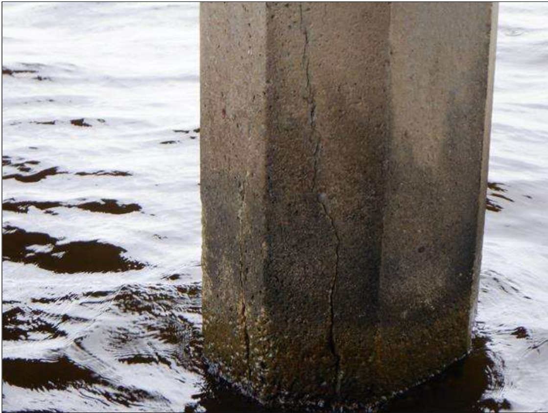
Bent 69 Pile 5: UW (PAR): H/L TO 1/8" CRACKS MULTIPLE FACES, FROM ABOVE THE HIGH WATER MARK DOWN THROUGH THE SPASH ZONE AND TAPERING TO HAIRLINE 1' TO 3' BELOW THE WATERLINE. SCALING TO 1" DEEP FROM WATERLINE TO MUDLINE.
