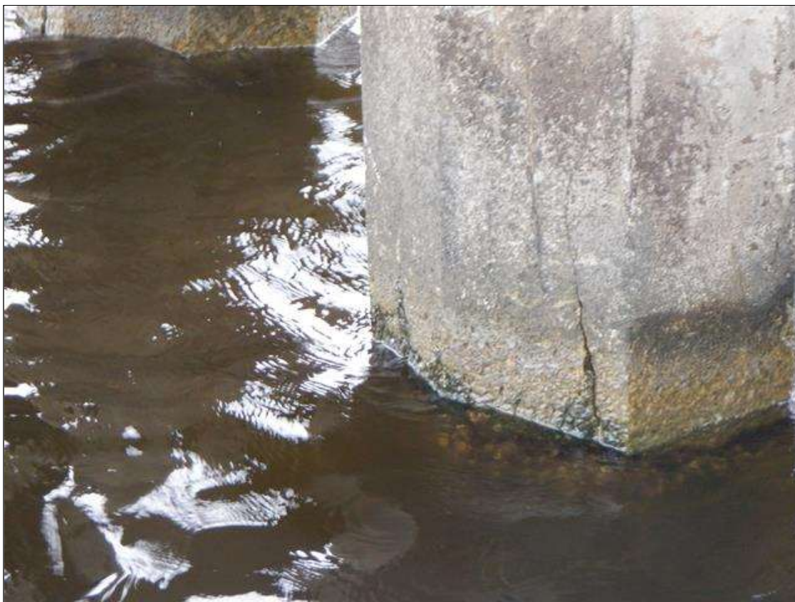
Bent 49 Saved Pile 4: UW (PAR): H/L TO 1/8" CRACKS MULTIPLE FACES, FROM ABOVE THE HIGH WATER MARK DOWN THROUGH THE SPASH ZONE AND TAPERING TO HAIRLINE 1' TO 3' BELOW THE WATERLINE. SCALING TO 1" DEEP FROM WATERLINE TO MUDLINE.
