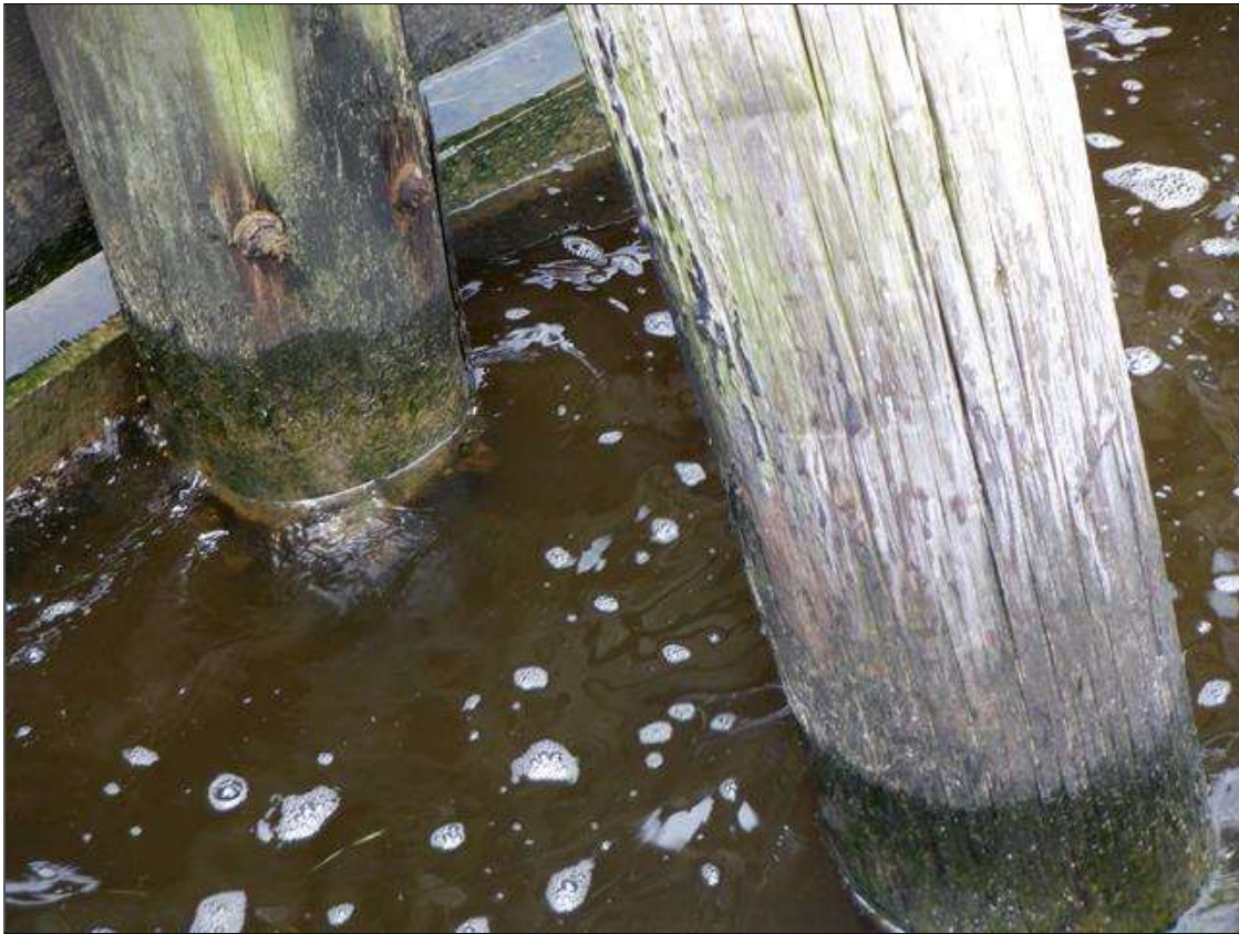
CHECKS TO 1/4" ON FENDER PILES
