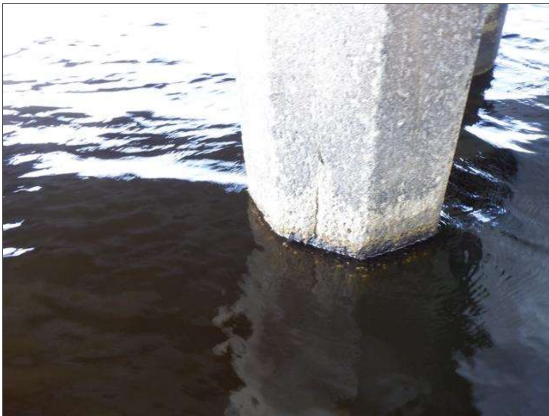
Bent 266 Pile 2: UW (PAR): H/L TO 1/8" CRACKS MULTIPLE FACES, FROM ABOVE THE HIGH WATER MARK DOWN THROUGH THE SPASH ZONE AND TAPERING TO HAIRLINE 1' TO 3' BELOW THE WATERLINE. SCALING TO 1" DEEP FROM WATERLINE TO MUDLINE.
