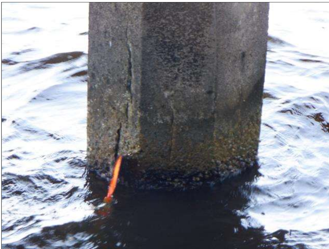
Bent 49 Saved Pile 5: UW (PAR): H/L TO 1/8" CRACKS MULTIPLE FACES, FROM ABOVE THE HIGH WATER MARK DOWN THROUGH THE SPASH ZONE AND TAPERING TO HAIRLINE 1' TO 3' BELOW THE WATERLINE. SCALING TO 1" DEEP FROM WATERLINE TO MUDLINE.
