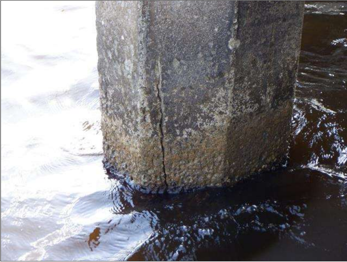
Bent 147 Pile 1: UW (PAR): H/L TO 1/8" CRACKS MULTIPLE FACES, FROM ABOVE THE HIGH WATER MARK DOWN THROUGH THE SPASH ZONE AND TAPERING TO HAIRLINE 1' TO 3' BELOW THE WATERLINE. SCALING TO 1" DEEP FROM WATERLINE TO MUDLINE.
