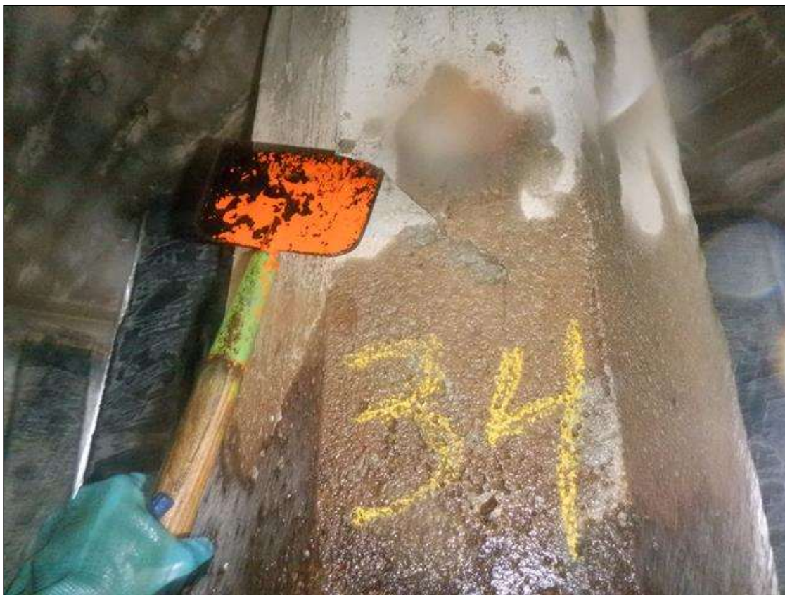
Bent 116 PIVOT Pile 34: U/W (PAR): CRACKED TO 1/8", DELAMINATED 1" TO 3" DEEP, MULTIPLE FACES, FROM CAP DOWN 4'. SCALING TO 1" DEEP FROM WATERLINE TO MUDLINE.
