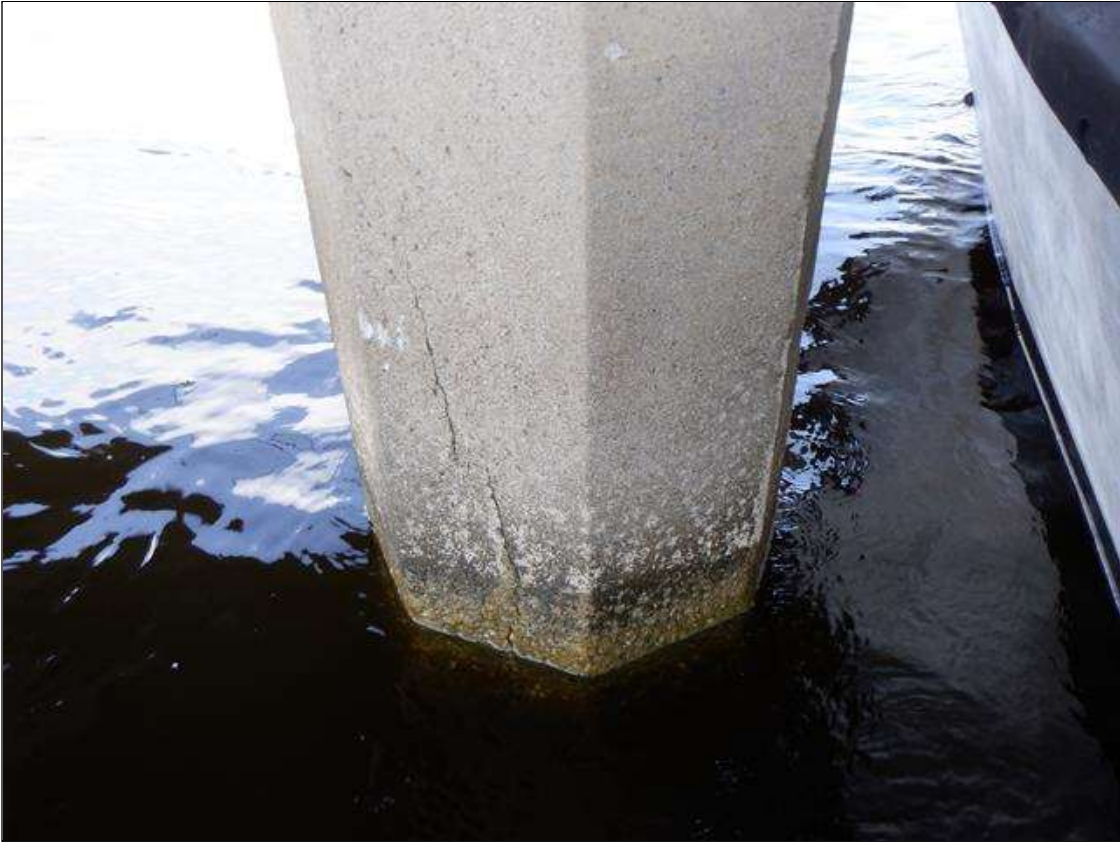
Bent 28 Saved Pile 2: UW (PAR): H/L TO 1/8" CRACKS MULTIPLE FACES, FROM ABOVE THE HIGH WATER MARK DOWN THROUGH THE SPASH ZONE AND TAPERING TO HAIRLINE 1' TO 3' BELOW THE WATERLINE. SCALING TO 1" DEEP FROM WATERLINE TO MUDLINE.
