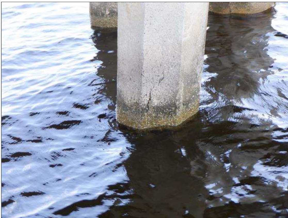
Bent 29 Saved Pile 4: UW (PAR): H/L TO 1/8" CRACKS MULTIPLE FACES, FROM ABOVE THE HIGH WATER MARK DOWN THROUGH THE SPASH ZONE AND TAPERING TO HAIRLINE 1' TO 3' BELOW THE WATERLINE. SCALING TO 1" DEEP FROM WATERLINE TO MUDLINE.
