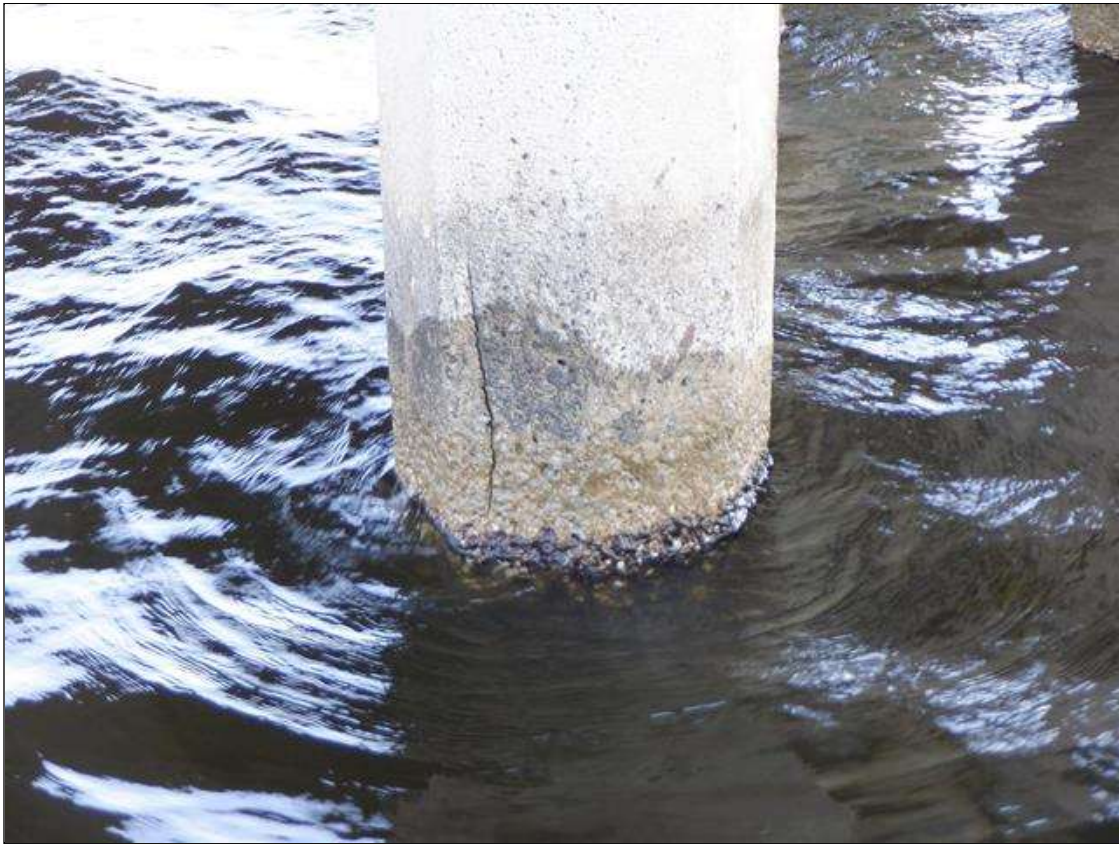
Bent 139 Pile 6: UW (PAR): H/L TO 1/8" CRACKS MULTIPLE FACES, FROM ABOVE THE HIGH WATER MARK DOWN THROUGH THE SPASH ZONE AND TAPERING TO HAIRLINE 1' TO 3' BELOW THE WATERLINE. SCALING TO 1" DEEP FROM WATERLINE TO MUDLINE.
