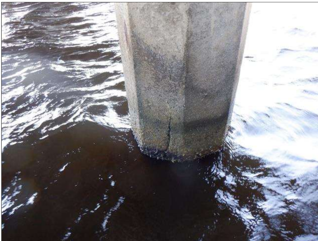
Bent 37 Saved Pile 5: UW (PAR): H/L TO 1/8" CRACKS MULTIPLE FACES, FROM ABOVE THE HIGH WATER MARK DOWN THROUGH THE SPASH ZONE AND TAPERING TO HAIRLINE 1' TO 3' BELOW THE WATERLINE. SCALING TO 1" DEEP FROM WATERLINE TO MUDLINE.
