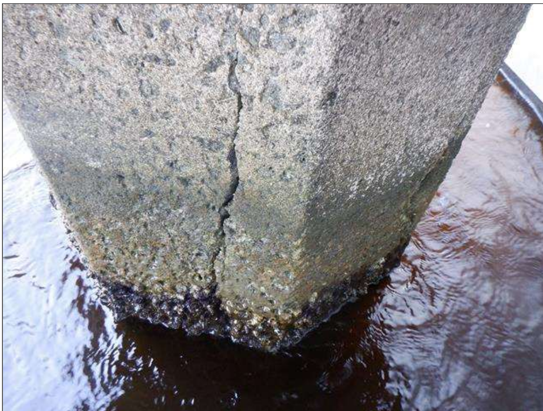
Bent 37 Saved Pile 6: UW (PAR): H/L TO 1/8" CRACKS MULTIPLE FACES, FROM ABOVE THE HIGH WATER MARK DOWN THROUGH THE SPASH ZONE AND TAPERING TO HAIRLINE 1' TO 3' BELOW THE WATERLINE. SCALING TO 1" DEEP FROM WATERLINE TO MUDLINE.
