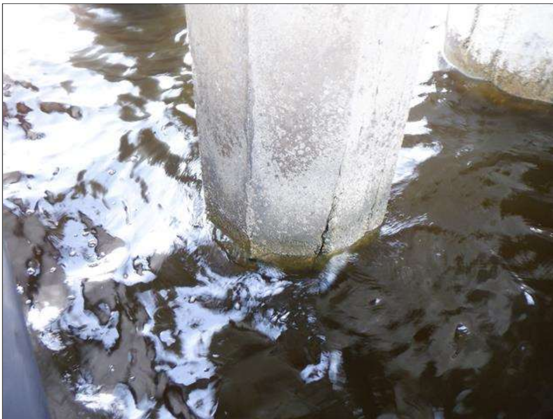
Bent 21 Saved Pile 5: UW (PAR): H/L TO 1/8" CRACKS MULTIPLE FACES, FROM ABOVE THE HIGH WATER MARK DOWN THROUGH THE SPASH ZONE AND TAPERING TO HAIRLINE 1' TO 3' BELOW THE WATERLINE. SCALING TO 1" DEEP FROM WATERLINE TO MUDLINE.
