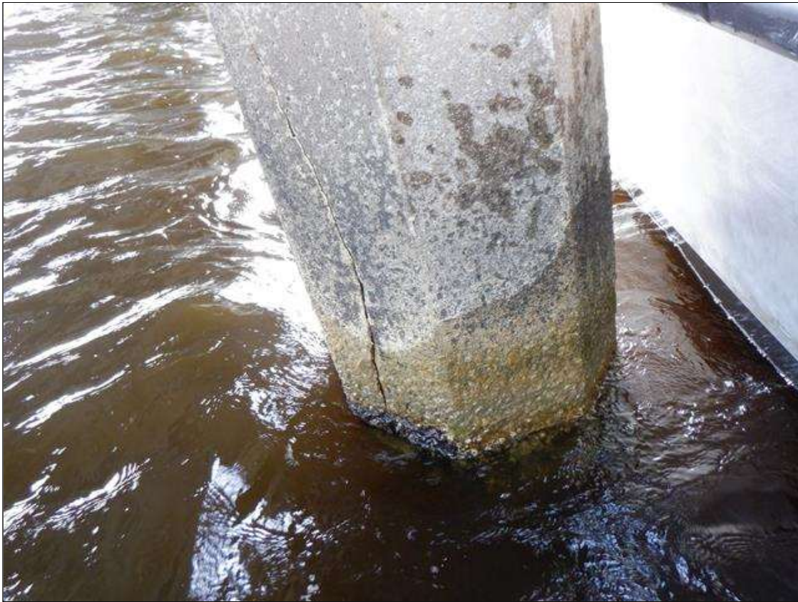
Bent 200 Pile 4: UW (PAR): H/L TO 1/8" CRACKS MULTIPLE FACES, FROM ABOVE THE HIGH WATER MARK DOWN THROUGH THE SPASH ZONE AND TAPERING TO HAIRLINE 1' TO 3' BELOW THE WATERLINE. SCALING TO 1" DEEP FROM WATERLINE TO MUDLINE.
