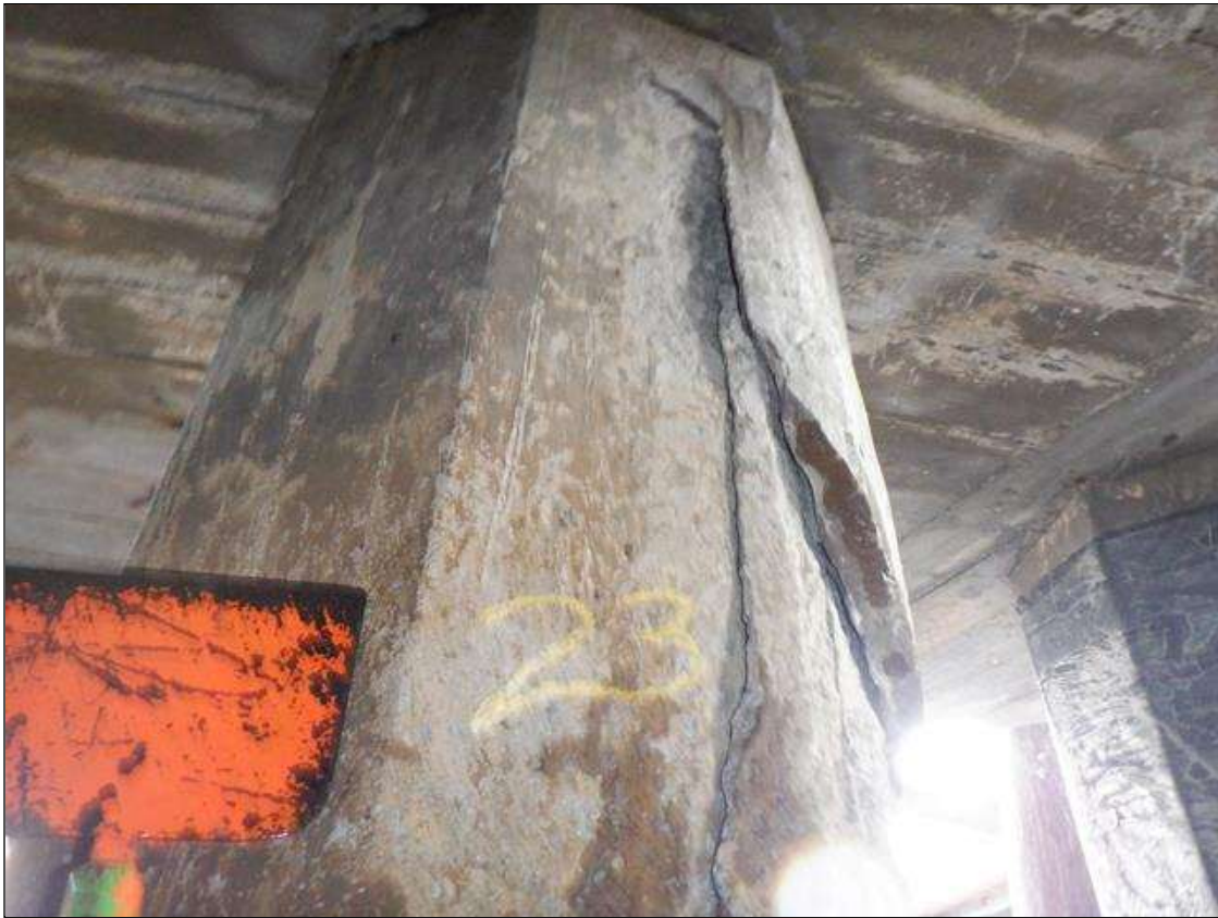
Bent 116 PIVOT Pile 23: U/W (PAR): CRACKED TO 1/8", DELAMINATED 1" TO 3" DEEP, MULTIPLE FACES, FROM CAP DOWN 4'. SCALING TO 1" DEEP FROM WATERLINE TO MUDLINE.
