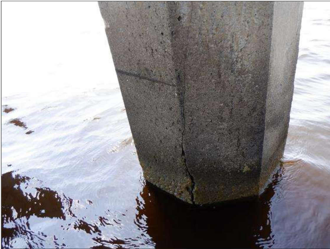
Bent 27 Saved Pile 4: UW (PAR): H/L TO 1/8" CRACKS MULTIPLE FACES, FROM ABOVE THE HIGH WATER MARK DOWN THROUGH THE SPASH ZONE AND TAPERING TO HAIRLINE 1' TO 3' BELOW THE WATERLINE. SCALING TO 1" DEEP FROM WATERLINE TO MUDLINE.
