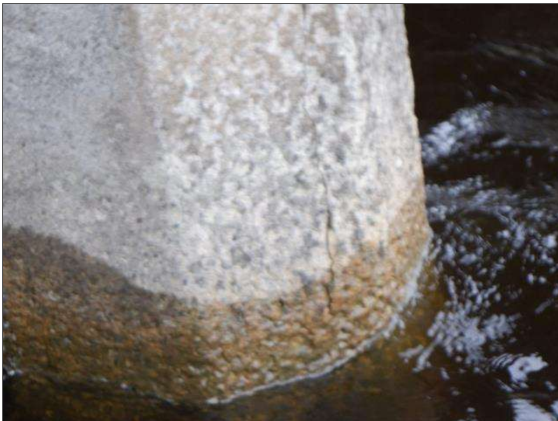
TYPICAL H/L TO 1/16" CRACKS
