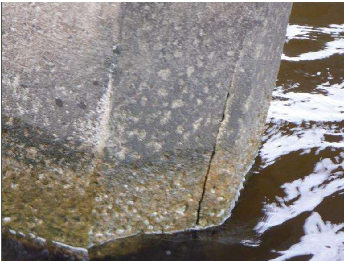
Bent 43 Saved Pile 4: UW (PAR): H/L TO 1/8" CRACKS MULTIPLE FACES, FROM ABOVE THE HIGH WATER MARK DOWN THROUGH THE SPASH ZONE AND TAPERING TO HAIRLINE 1' TO 3' BELOW THE WATERLINE. SCALING TO 1" DEEP FROM WATERLINE TO MUDLINE.
