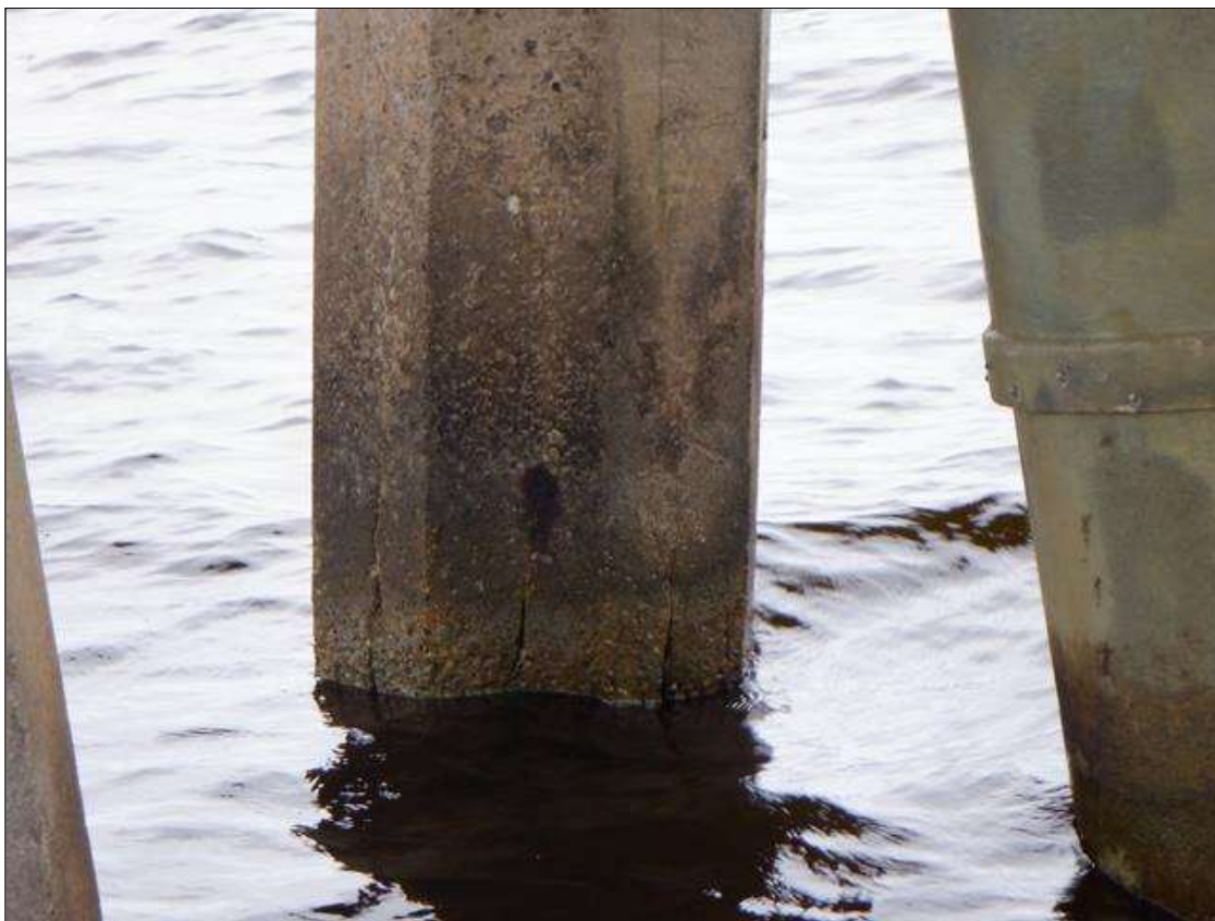
Bent 65 Pile 5: UW (PAR): H/L TO 1/8" CRACKS MULTIPLE FACES, FROM ABOVE THE HIGH WATER MARK DOWN THROUGH THE SPASH ZONE AND TAPERING TO HAIRLINE 1' TO 3' BELOW THE WATERLINE. SCALING TO 1" DEEP FROM WATERLINE TO MUDLINE.
