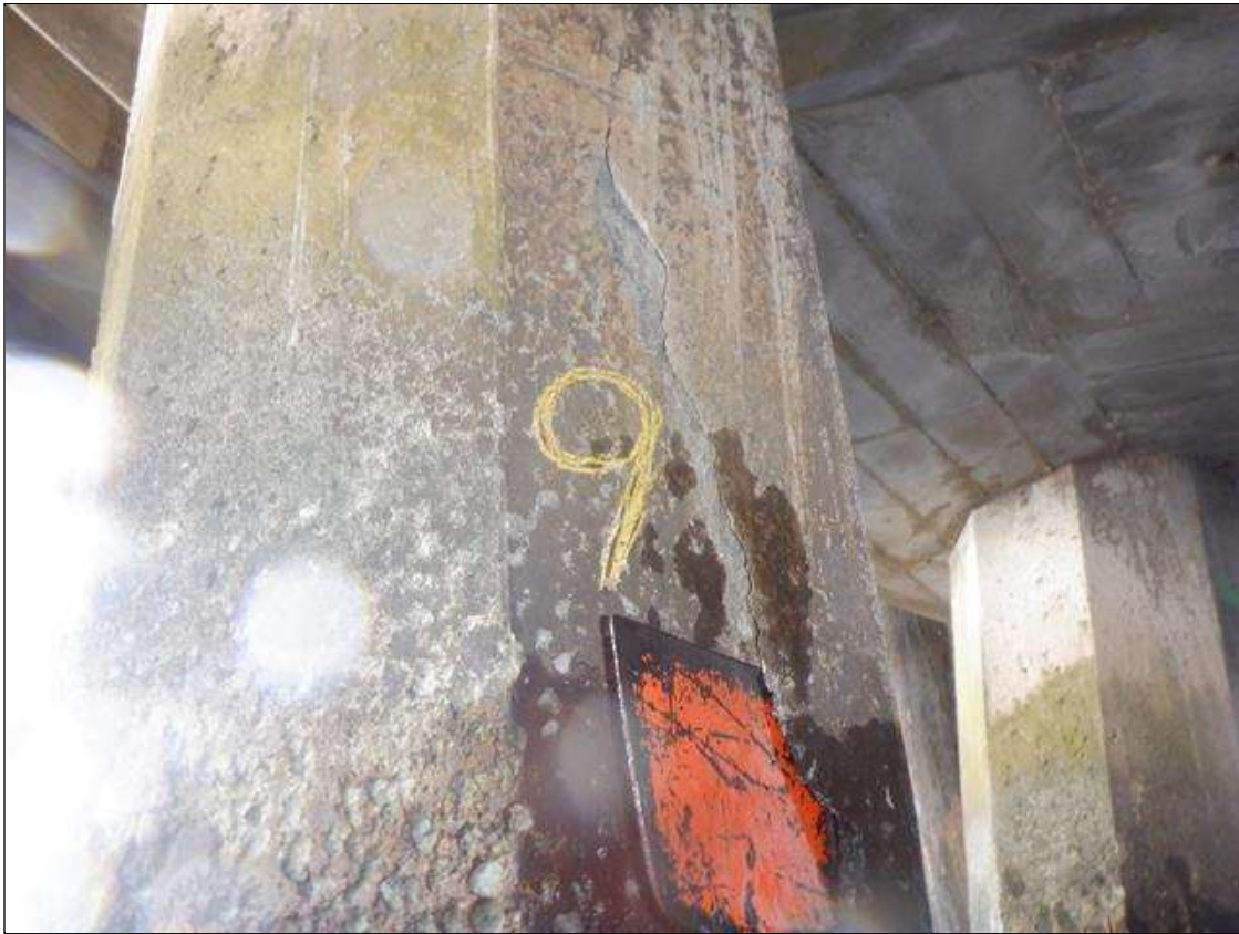
Bent 116 PIVOT Pile 9: U/W (PAR): CRACKED TO 1/8", DELAMINATED 1" TO 3" DEEP, MULTIPLE FACES, FROM CAP DOWN 4'. SCALING TO 1" DEEP FROM WATERLINE TO MUDLINE.
