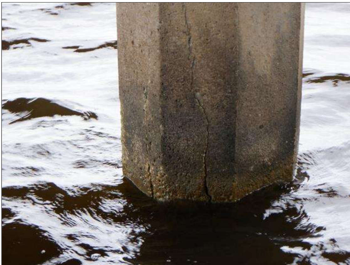
Bent 191 Pile 1: UW (PAR): H/L TO 1/8" CRACKS MULTIPLE FACES, FROM ABOVE THE HIGH WATER MARK DOWN THROUGH THE SPASH ZONE AND TAPERING TO HAIRLINE 1' TO 3' BELOW THE WATERLINE. SCALING TO 1" DEEP FROM WATERLINE TO MUDLINE.
