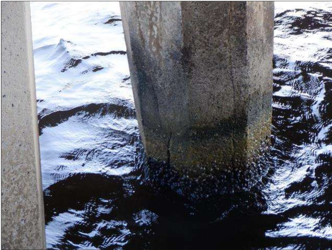
Bent 41 Saved Pile 4: UW (PAR): H/L TO 1/8" CRACKS MULTIPLE FACES, FROM ABOVE THE HIGH WATER MARK DOWN THROUGH THE SPASH ZONE AND TAPERING TO HAIRLINE 1' TO 3' BELOW THE WATERLINE. SCALING TO 1" DEEP FROM WATERLINE TO MUDLINE.
