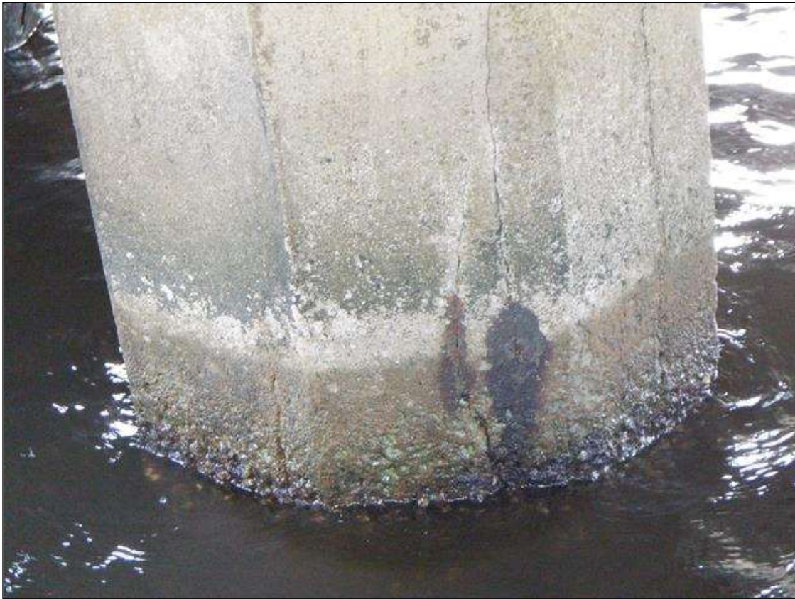
Bent 115 REST PIER 1 Pile 5: UW (PAR): H/L TO 1/8" CRACKS MULTIPLE FACES, FROM ABOVE THE HIGH WATER MARK DOWN THROUGH THE SPASH ZONE AND TAPERING TO HAIRLINE 1' TO 3' BELOW THE WATERLINE. SCALING TO 1" DEEP FROM WATERLINE TO MUDLINE.
