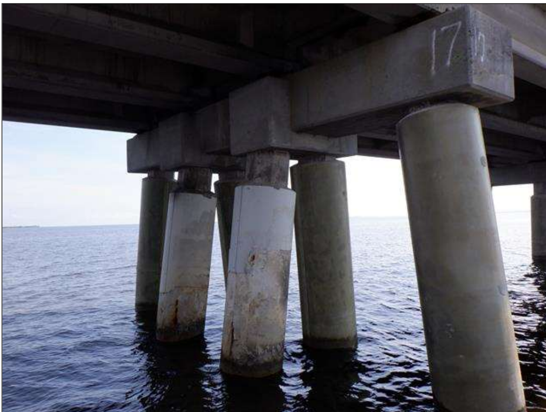
BENT 17 ALL PILES JACKETED, P-2 & P-4 JACKETES ARE IN POOR CONDITION
