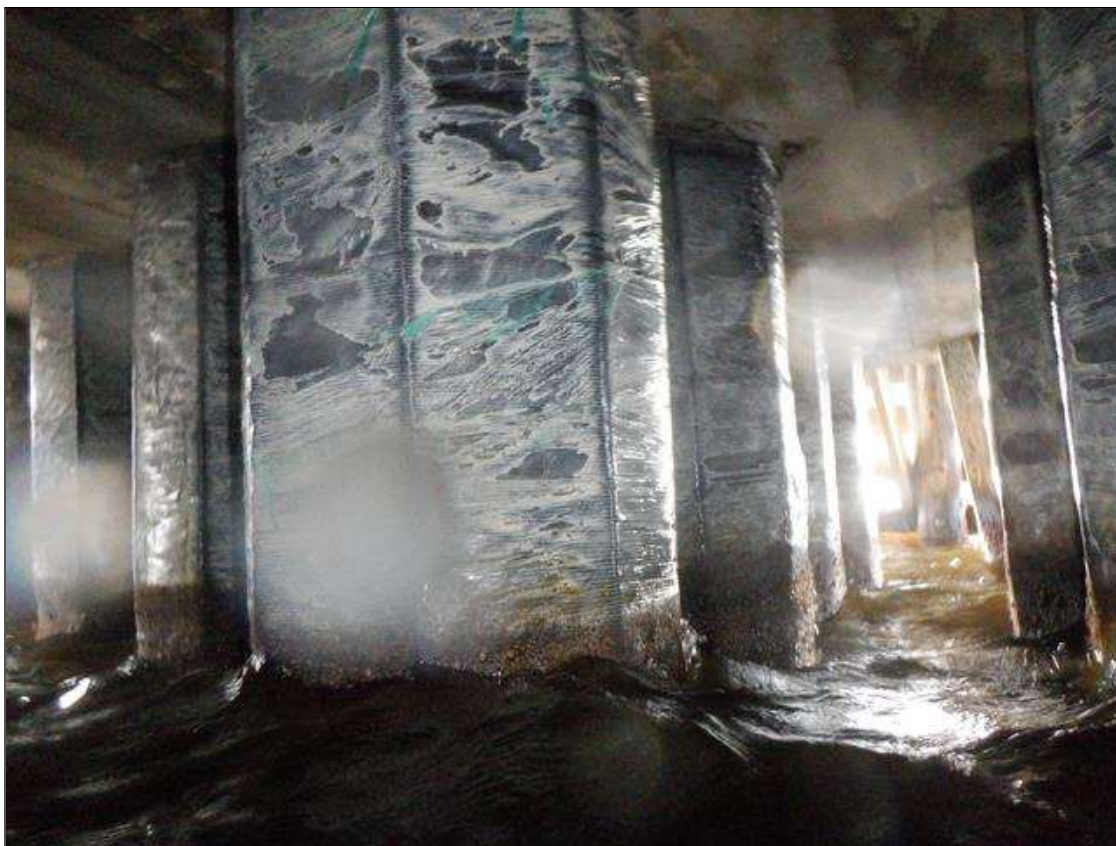
REPAIRED PIVOT PIER PILES
