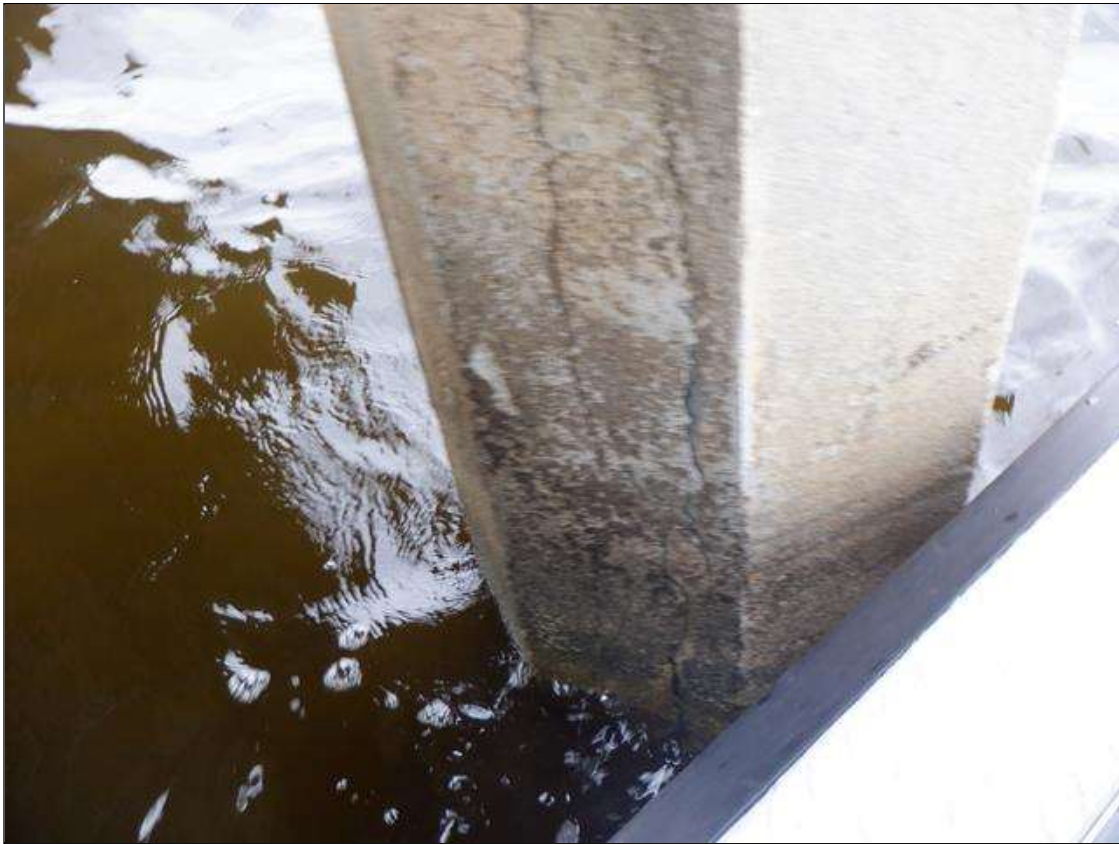
Bent 65 Pile 6: UW (PAR): H/L TO 1/8" CRACKS MULTIPLE FACES, FROM ABOVE THE HIGH WATER MARK DOWN THROUGH THE SPASH ZONE AND TAPERING TO HAIRLINE 1' TO 3' BELOW THE WATERLINE. SCALING TO 1" DEEP FROM WATERLINE TO MUDLINE.
