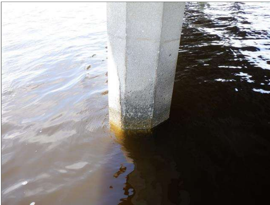
Bent 19 Saved Pile 4: UW (PAR): H/L TO 1/8" CRACKS MULTIPLE FACES, FROM ABOVE THE HIGH WATER MARK DOWN THROUGH THE SPASH ZONE AND TAPERING TO HAIRLINE 1' TO 3' BELOW THE WATERLINE. SCALING TO 1" DEEP FROM WATERLINE TO MUDLINE.
