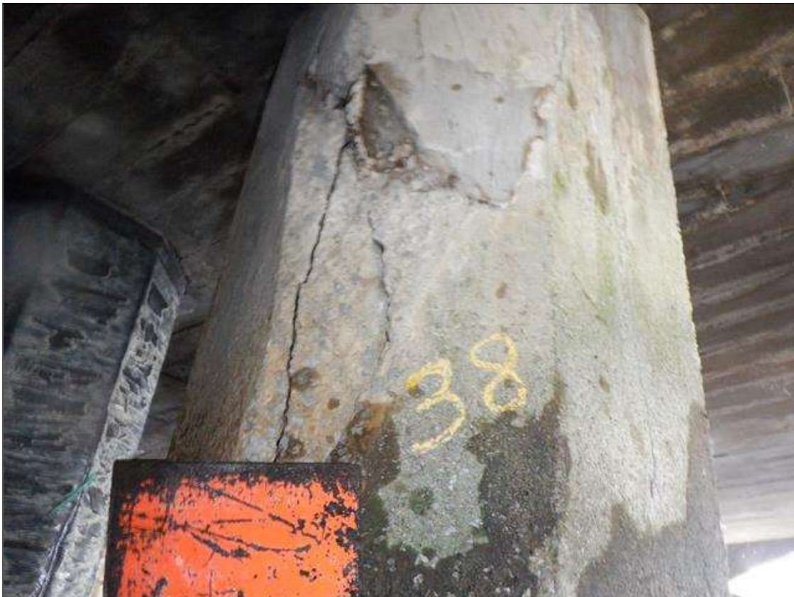
Bent 116 PIVOT Pile 38: U/W (PAR): CRACKED TO 1/8", DELAMINATED 1" TO 3" DEEP, MULTIPLE FACES, FROM CAP DOWN 4'. SCALING TO 1" DEEP FROM WATERLINE TO MUDLINE.
