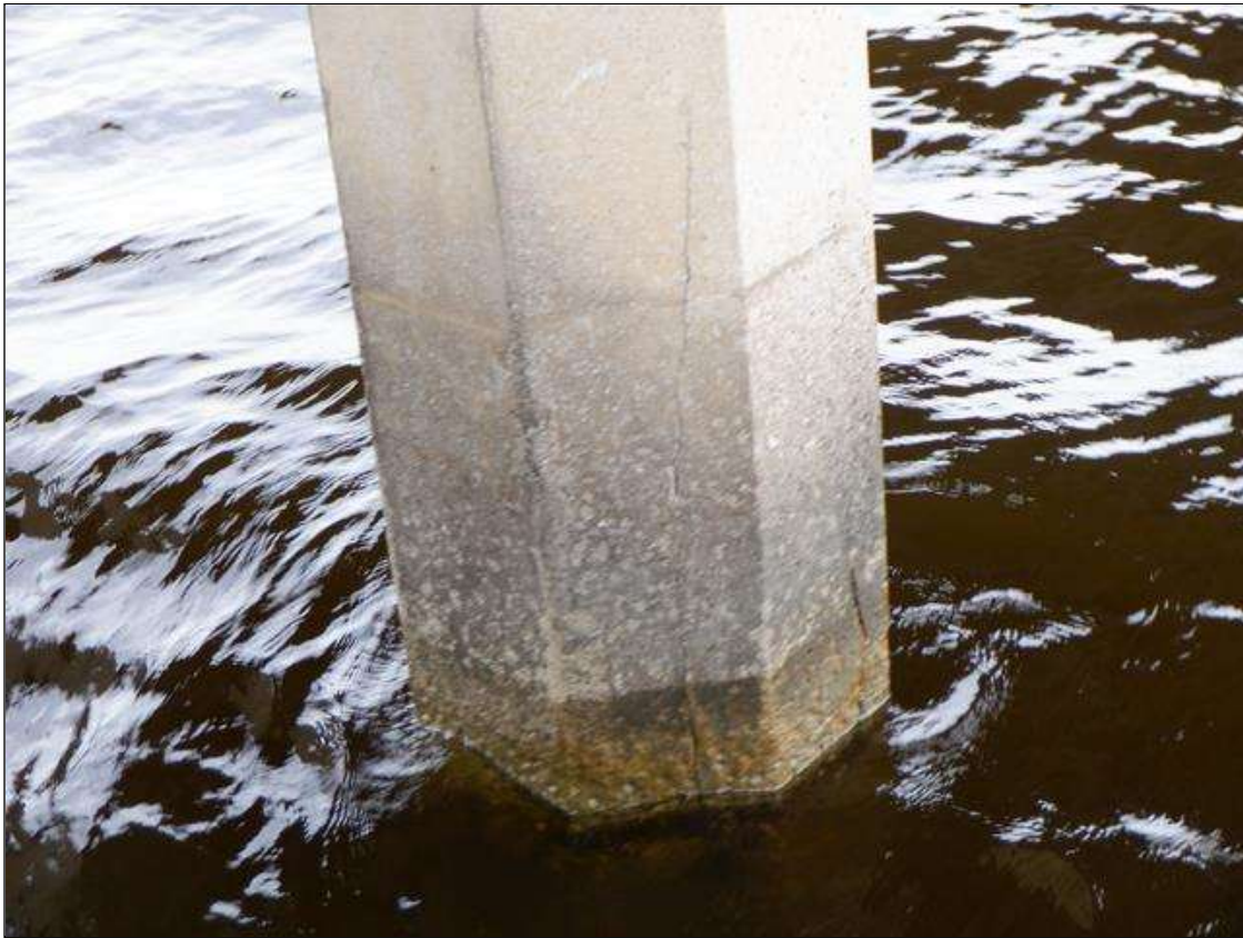
Bent 46 Saved Pile 2: UW (PAR): H/L TO 1/8" CRACKS MULTIPLE FACES, FROM ABOVE THE HIGH WATER MARK DOWN THROUGH THE SPASH ZONE AND TAPERING TO HAIRLINE 1' TO 3' BELOW THE WATERLINE. SCALING TO 1" DEEP FROM WATERLINE TO MUDLINE.
