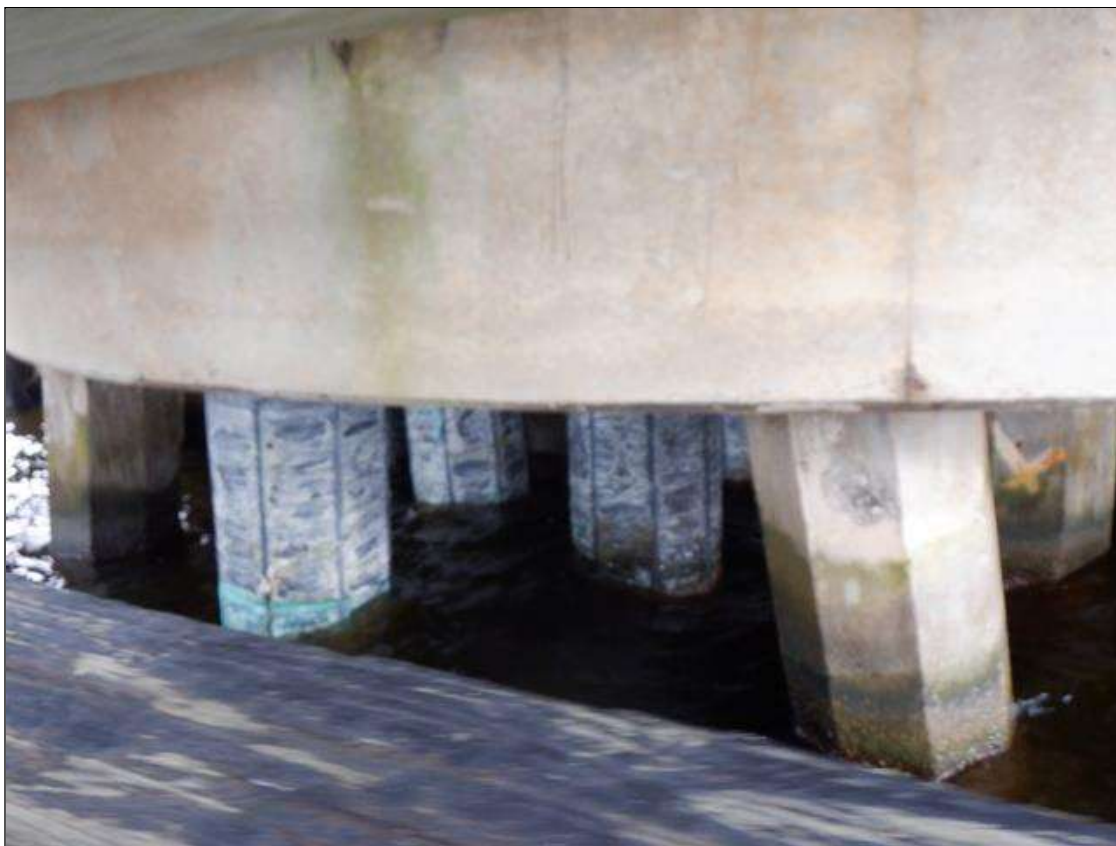
PIVOT BENT AND PILES
