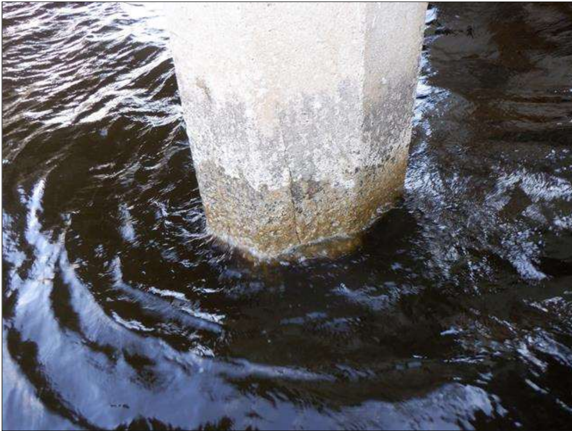
Bent 127 Pile 6: UW (PAR): H/L TO 1/8" CRACKS MULTIPLE FACES, FROM ABOVE THE HIGH WATER MARK DOWN THROUGH THE SPASH ZONE AND TAPERING TO HAIRLINE 1' TO 3' BELOW THE WATERLINE. SCALING TO 1" DEEP FROM WATERLINE TO MUDLINE.
