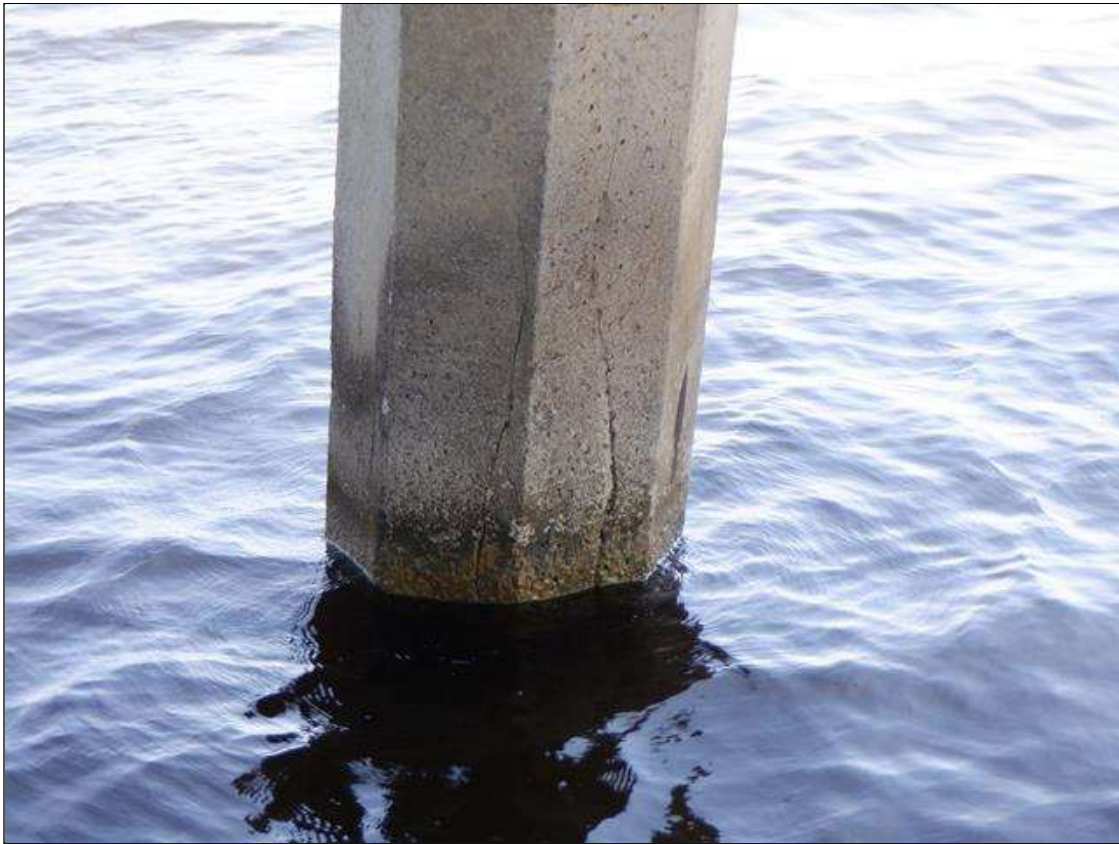
Bent 27 Saved Pile 1: UW (PAR): H/L TO 1/8" CRACKS MULTIPLE FACES, FROM ABOVE THE HIGH WATER MARK DOWN THROUGH THE SPASH ZONE AND TAPERING TO HAIRLINE 1' TO 3' BELOW THE WATERLINE. SCALING TO 1" DEEP FROM WATERLINE TO MUDLINE.
