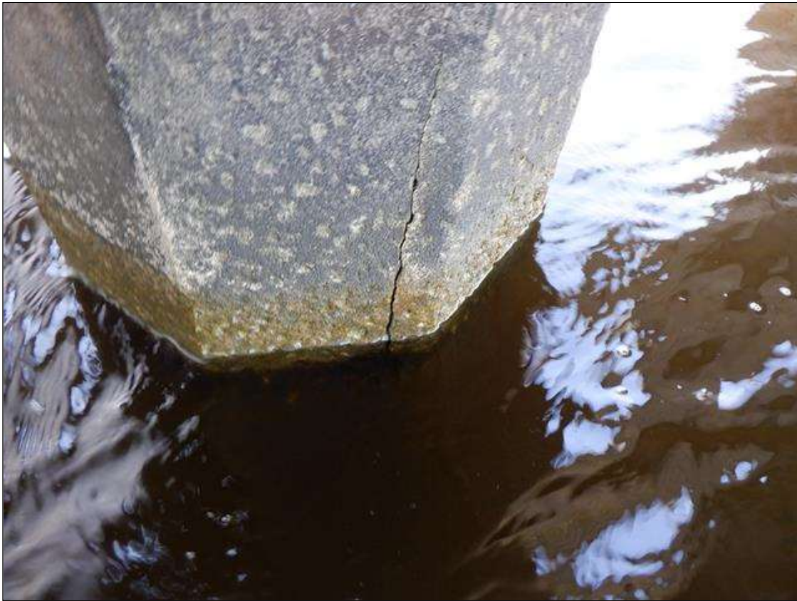
Bent 40 Saved Pile 4: UW (PAR): H/L TO 1/8" CRACKS MULTIPLE FACES, FROM ABOVE THE HIGH WATER MARK DOWN THROUGH THE SPASH ZONE AND TAPERING TO HAIRLINE 1' TO 3' BELOW THE WATERLINE. SCALING TO 1" DEEP FROM WATERLINE TO MUDLINE.
