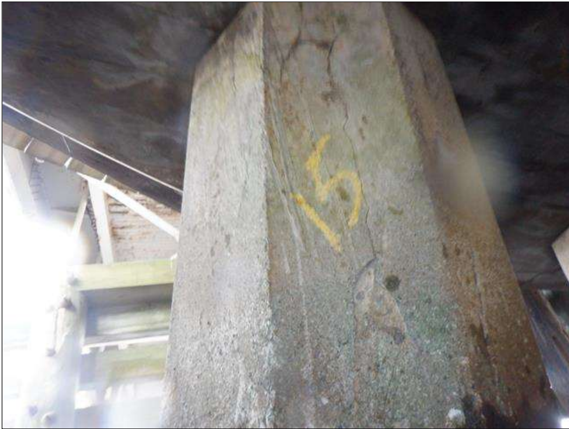
Bent 116 PIVOT Pile 15: U/W (PAR): CRACKED TO 1/8", DELAMINATED 1" TO 3" DEEP, MULTIPLE FACES, FROM CAP DOWN 4'. SCALING TO 1" DEEP FROM WATERLINE TO MUDLINE.
