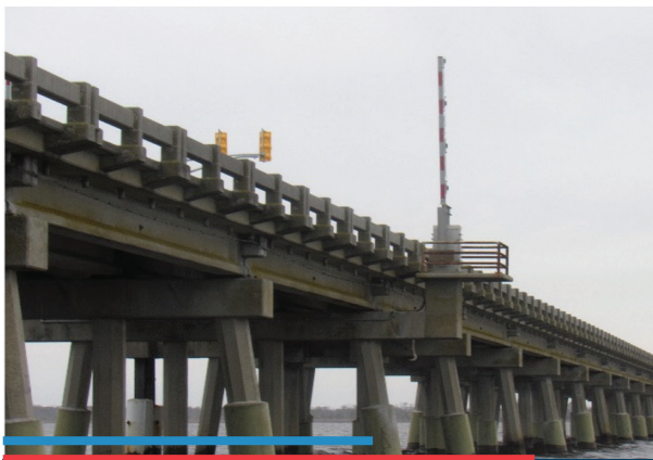
Figure 5: Rehabilitation of Bridge Included Pile Jacketing
