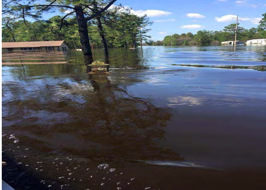
Figure 5B-5. Hurricane Florence flooding at the NC Forest Service Duplin/Pender Zone site (2018)
