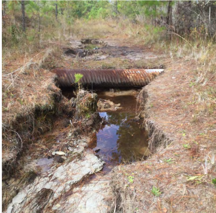
Figure 5B-7: 2018 Hurricane damaged road at Hog Branch Ponds Plant Conservation Preserve, Brunswick County
