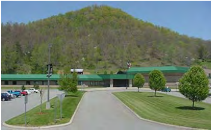
Figure 3: Robbinsville High and Middle School building
