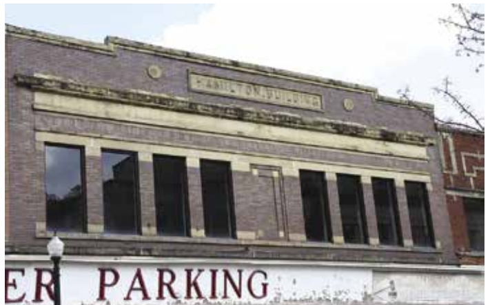
f8.4 Williamson, West Virginia transformed a vacant downtown building into a parking structure.
