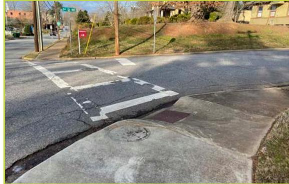
*The sidewalk transition to curb ramp is sometimes narrow and does not meet accessibility standards.*
