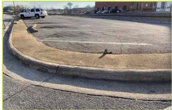
*Sidewalk lacks curb ramps and does not meet ADA-accessibility standards.*
