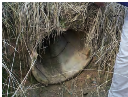
Example: Crossline Pipe Damaged
