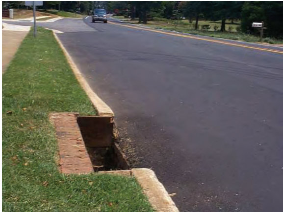
Examples: Inlets Damaged / Missing
