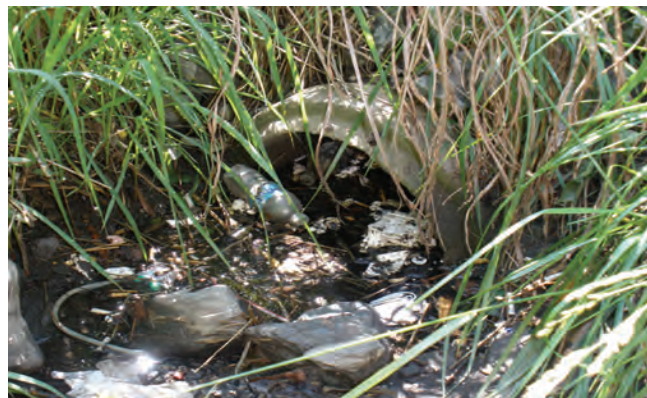
Examples: Crossline Pipes Blocked
