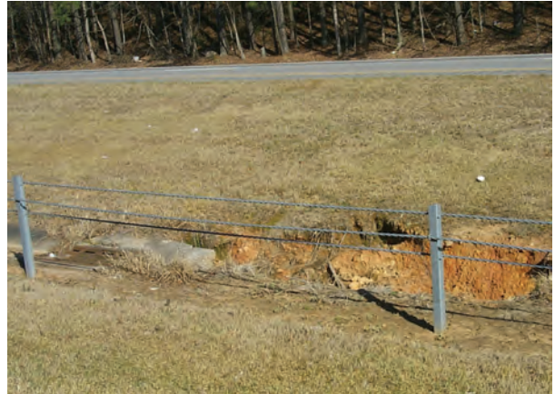
Examples: Inlets Damaged / Missing
