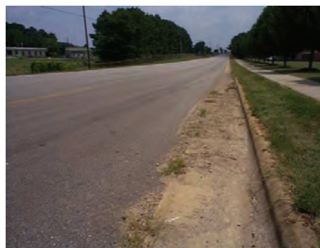
Examples: Gutters Blocked
