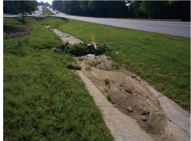
Examples: Lateral Ditches — Blocked
