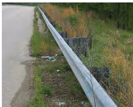
Examples: Gutters Blocked
