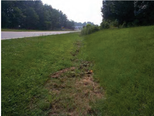
Examples: Lateral Ditches — Blocked
