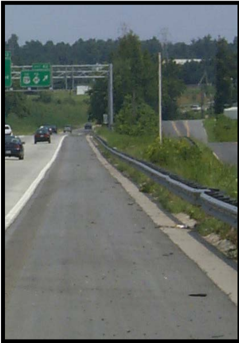
Maintenance Condition Survey
