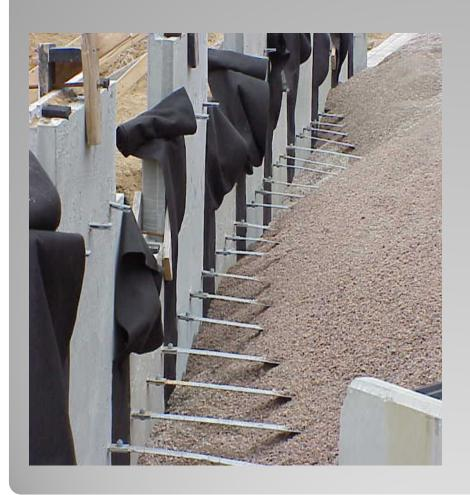
Utilizes straps that are bolted to panels and are backfilled with various stone sizes and or screened backfill.
