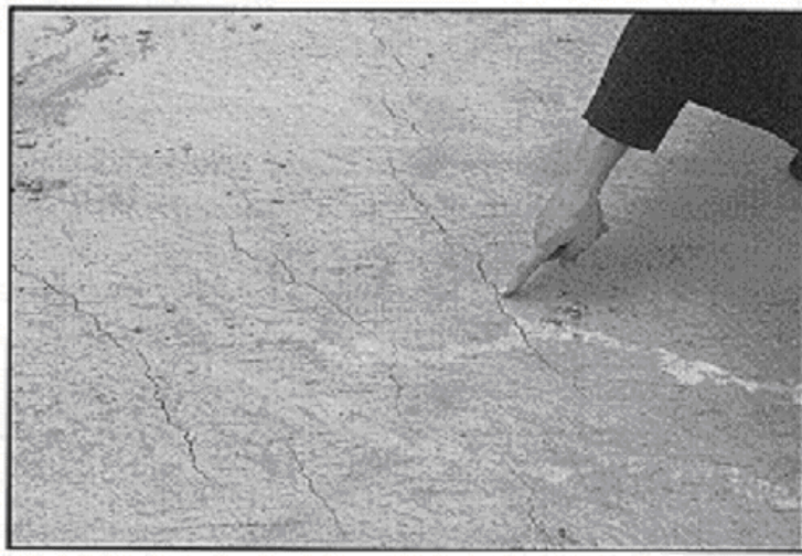
Plastic Shrinkage Cracks
