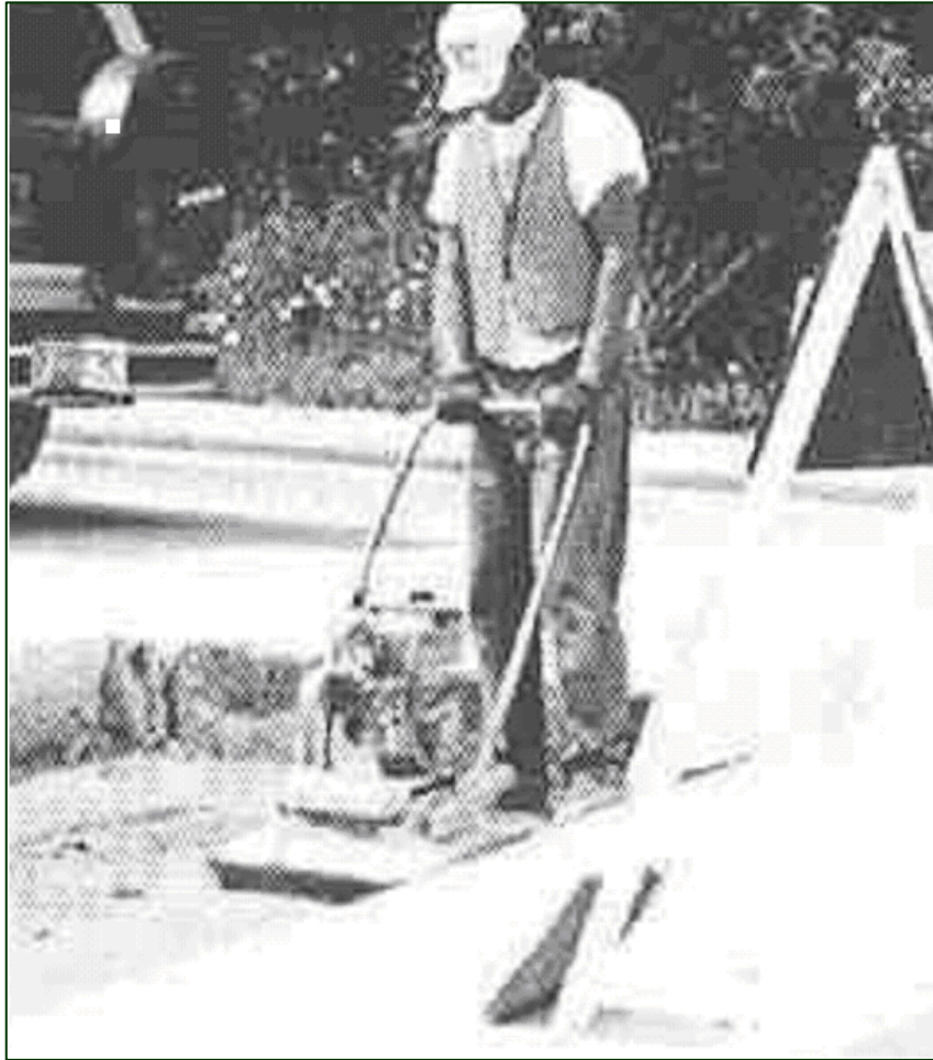
REPAIRING THE BASE LAYER
