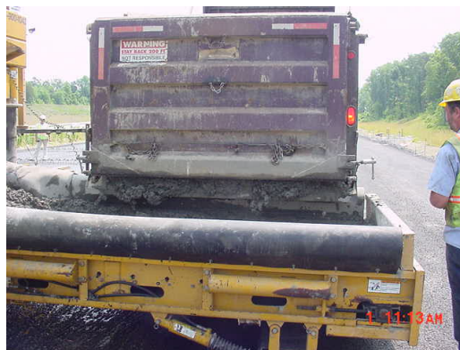
The spreader belt can be dangerous.
