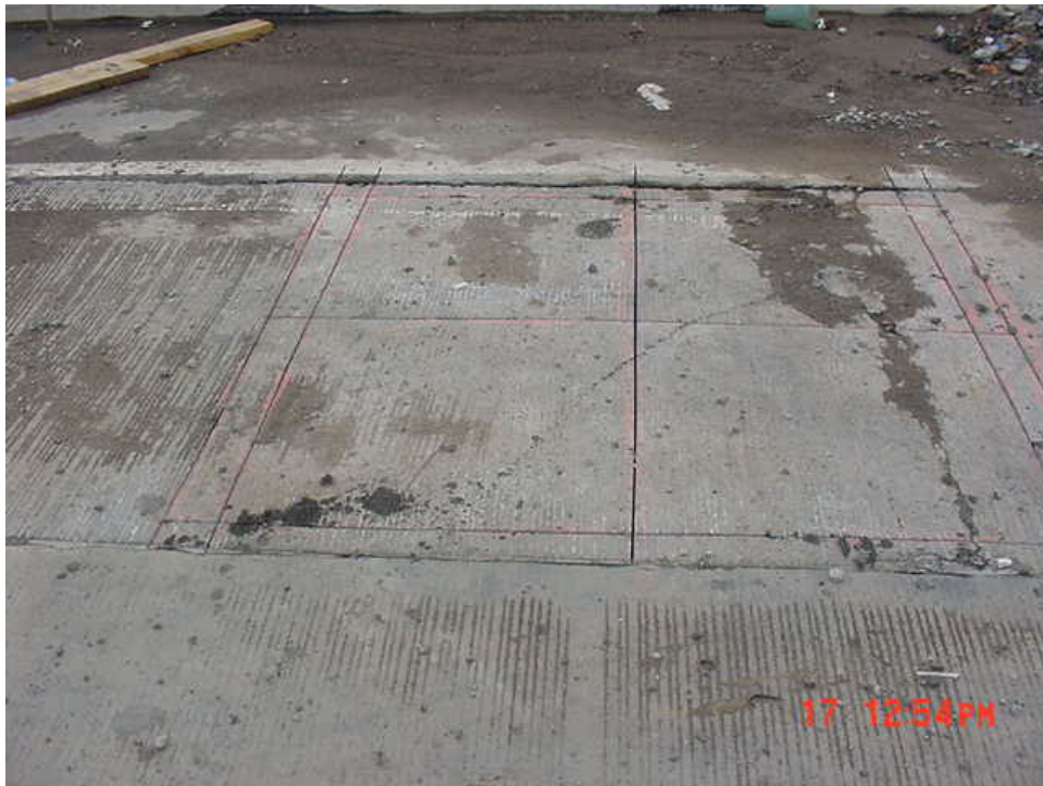
THE SAW CUTS FOR THE LIFTOUT METHOD
