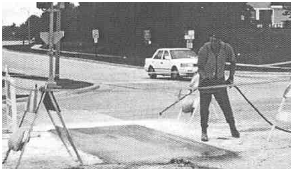
Protect the Repair From Rapid Evaporation
