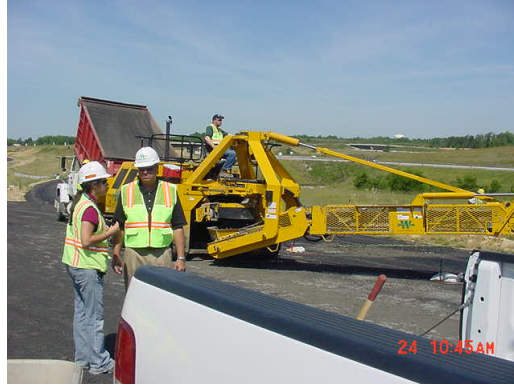
Spreader belts can be a danger
