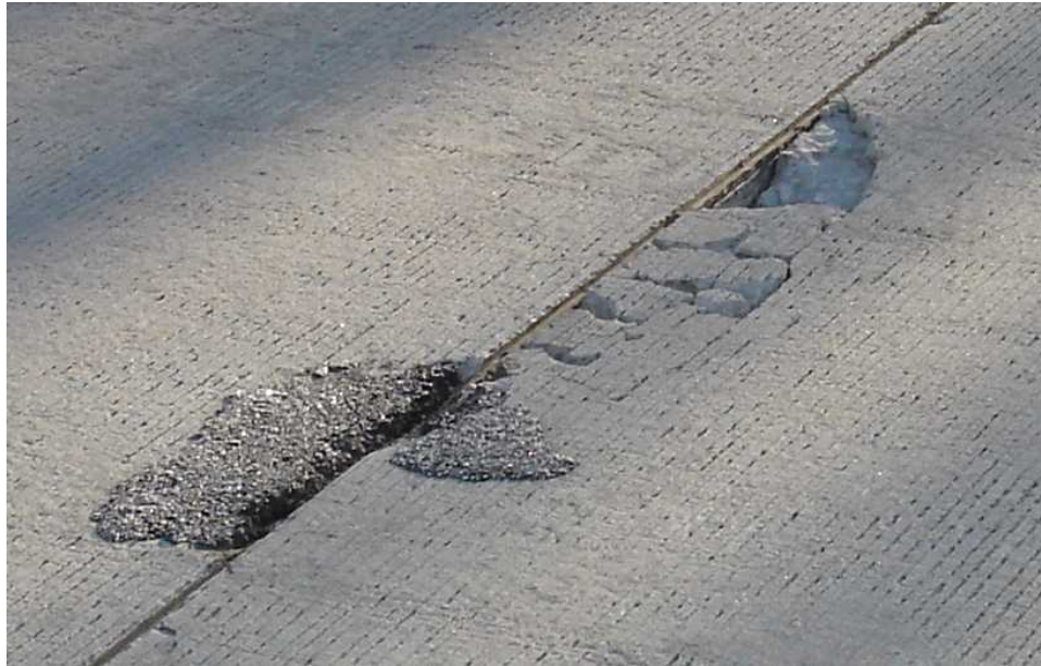
SPALL AT TRANSVERSE JOINT
