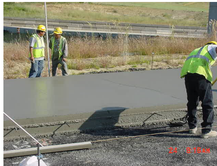
Stringlines can be a tripping hazard
