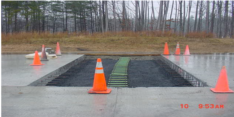
PLACING LOAD TRANSFER DEVICE
