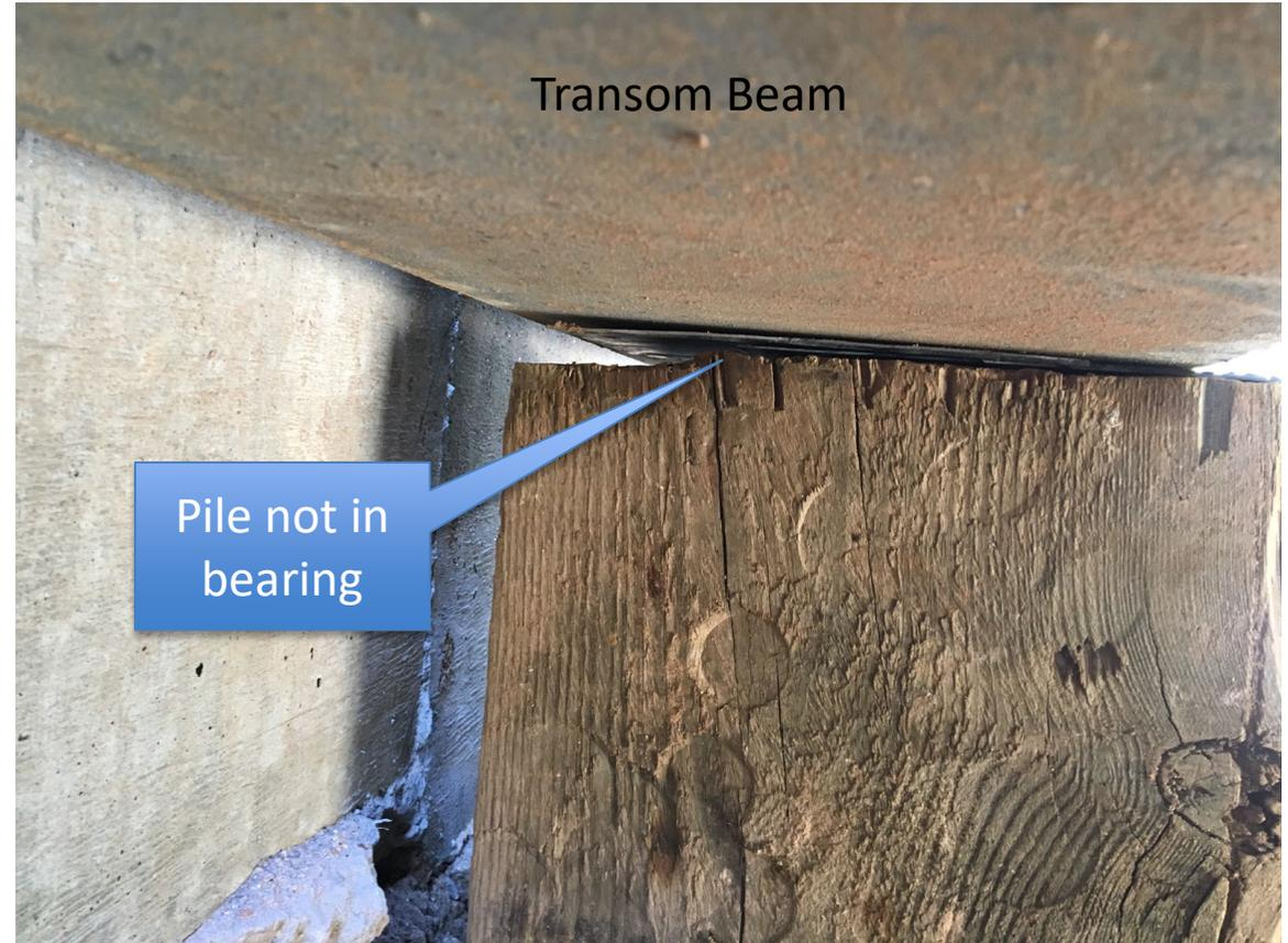
Bolster detail showing timber on H-Pile
