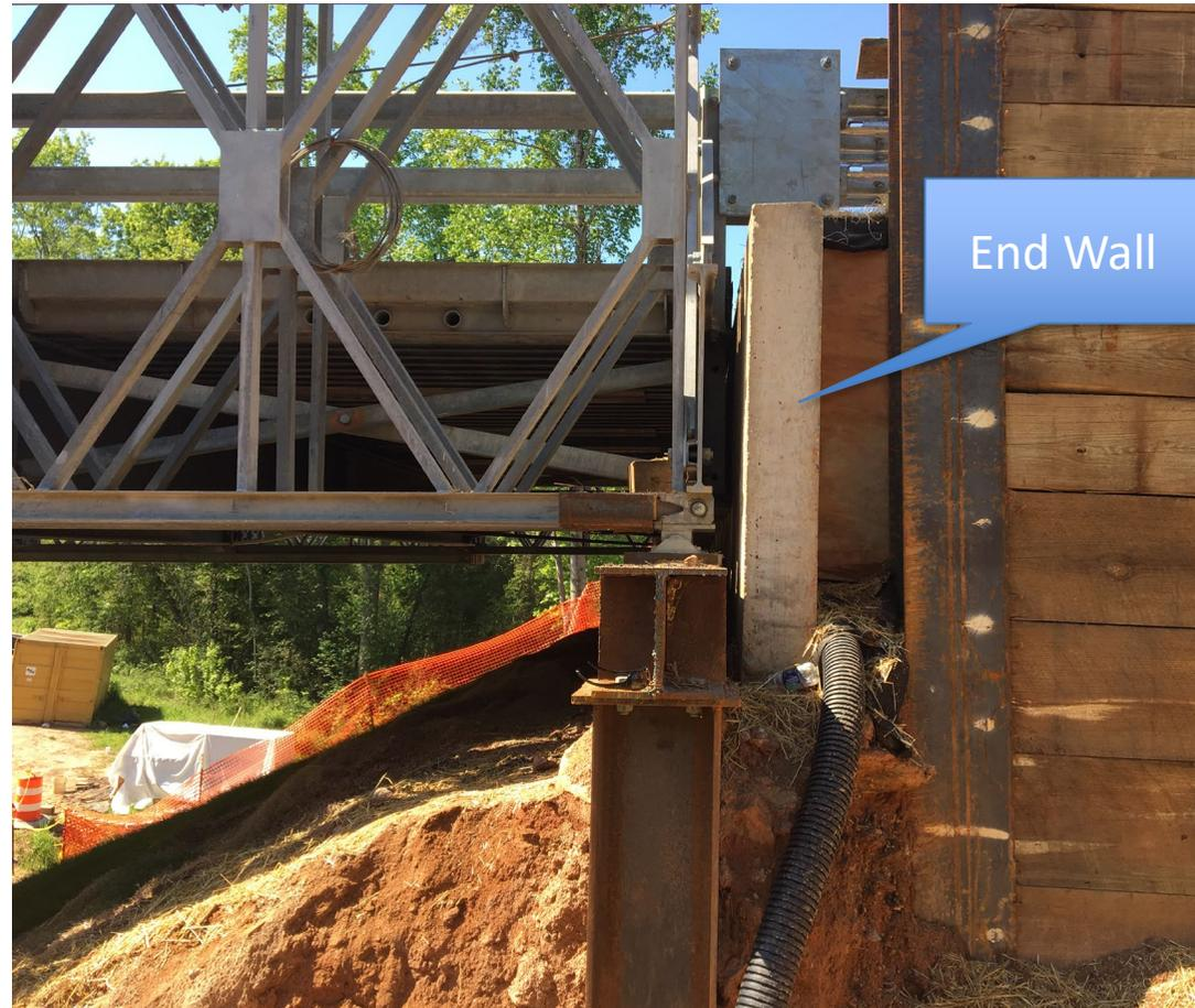
Verify clearance from the end wall to the transom beam. Typically the transom beam is coped.
