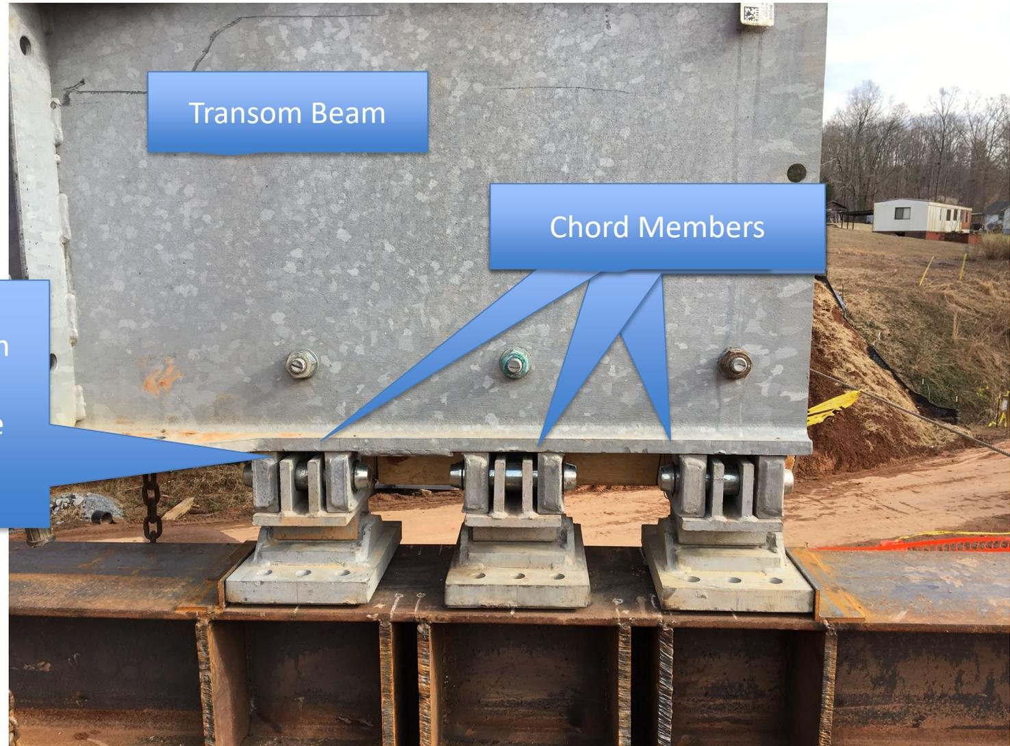
If the bottom flange of the transom beam is not bearing on the chord members it could potentially place panel bolts in shear
