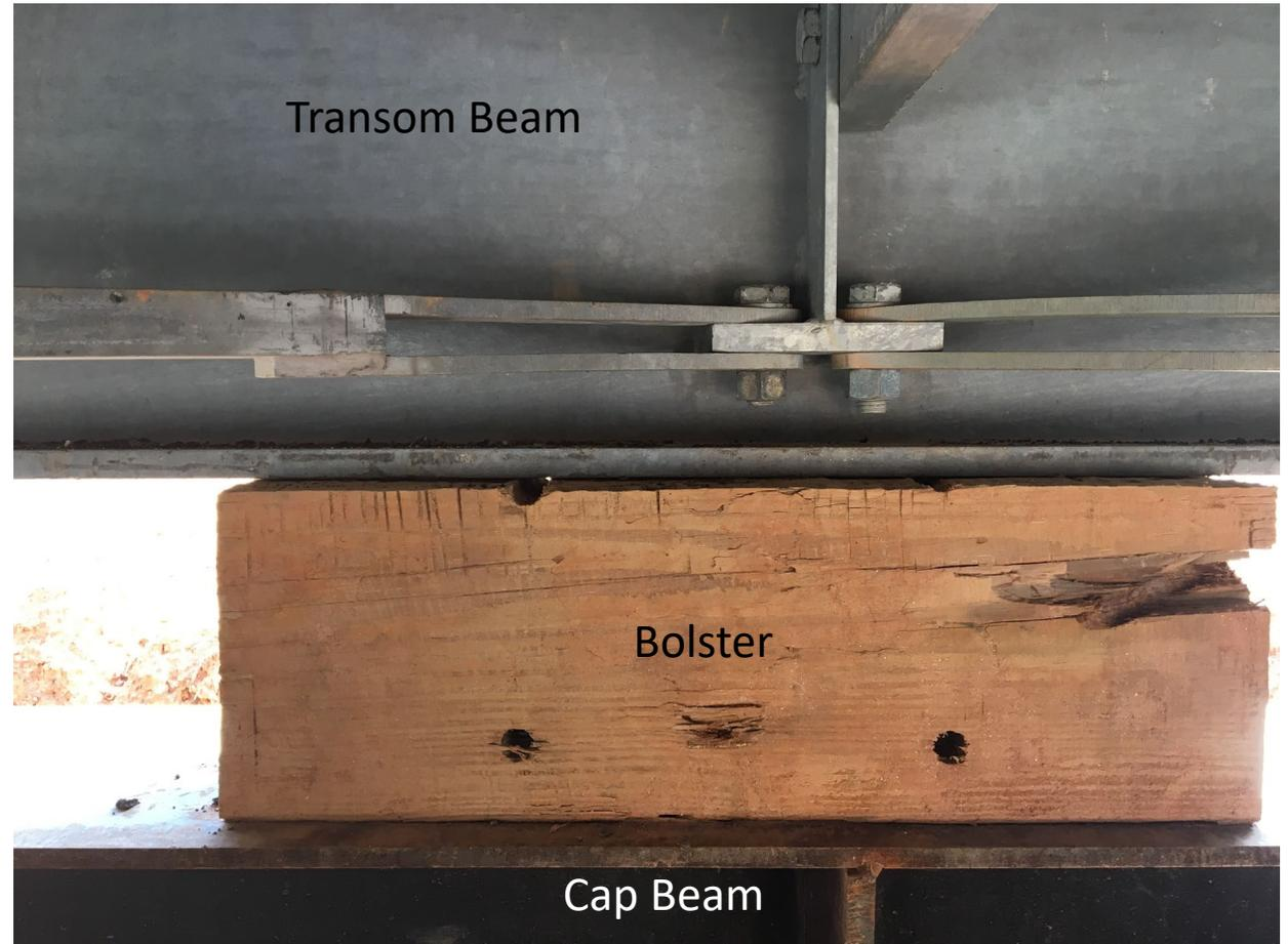
Bolster not attached to the cap beam
