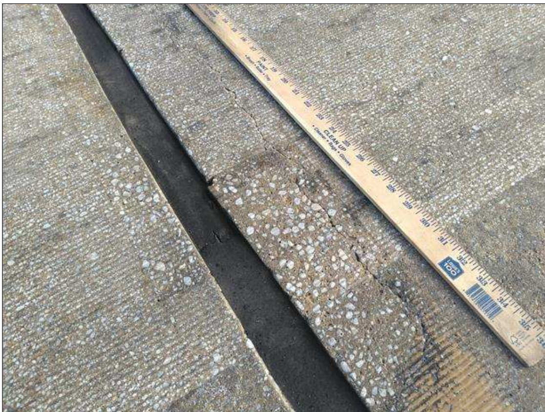
Span 203 Expansion Joint Bent 202: RIGHT LANE ALONG JOINT, PATCHED AREA (UP TO 10FEET X 4 INCHES). 0.06 INCH CRACK AND DELAMINATION AT PATCHES
