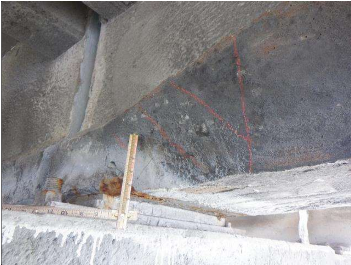
Span 106 Beam 3: NORTH FACE AT BENT 106, DELAMINATION/FAILED PATCH (12 INCHES X 8 INCHES X 2 INCHES)
