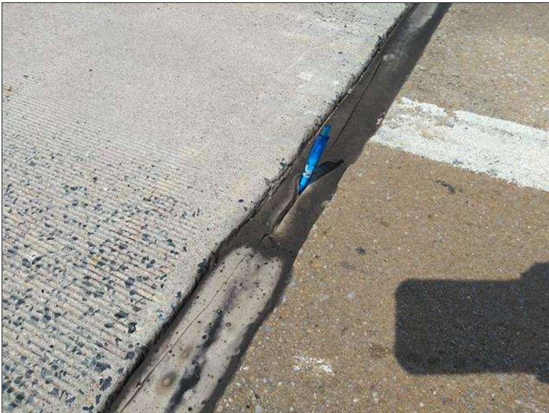
Span 155 Expansion Joint Bent 154: AT BENT 154, CRACKING FULL DEPTH THROUGHOUT
