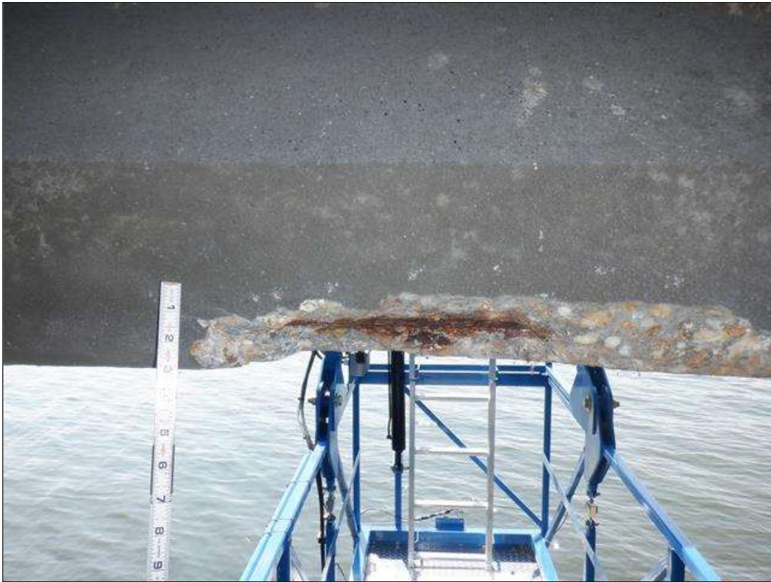
Span 161 Beam 4: (PAR) BOTTOM FLANGE NORTH FACE AT 3 FEET FROM BENT 160, SPALL (32 INCHES LONG X 5 INCHES WIDE X UP TO 2 INCHES DEEP) WITH EXPOSED RUSTED STRANDS (10 PERCENT SECTION LOSS)
