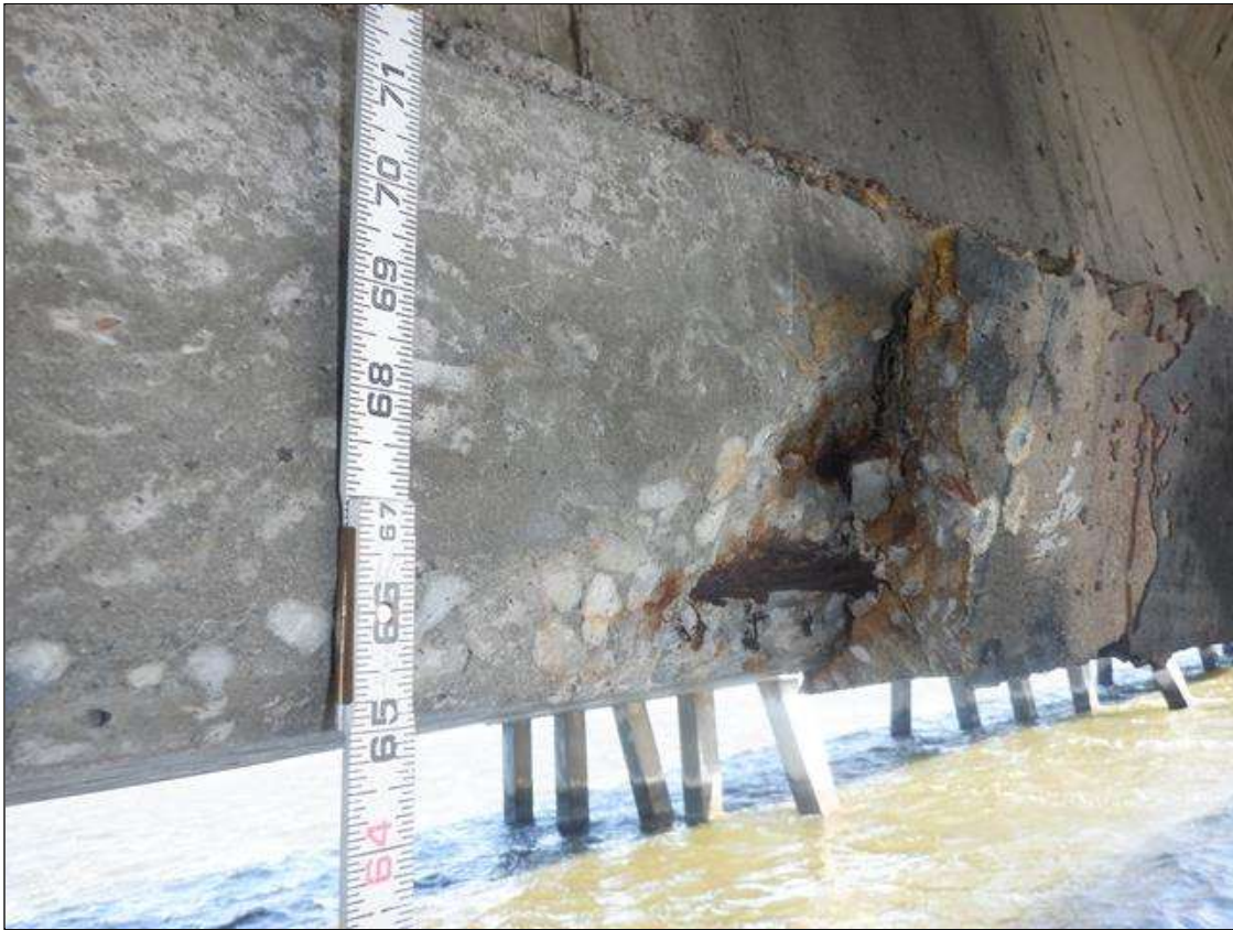
Span 100 Beam 1: (PAR) SOUTH FACE OF BOTTOM FLANGE AT 8 FEET FROM BENT 99, FAILED PATCHED ARE. (48 INCHES X 7 INCHES X UP TO 2 INCHES DEEP)
