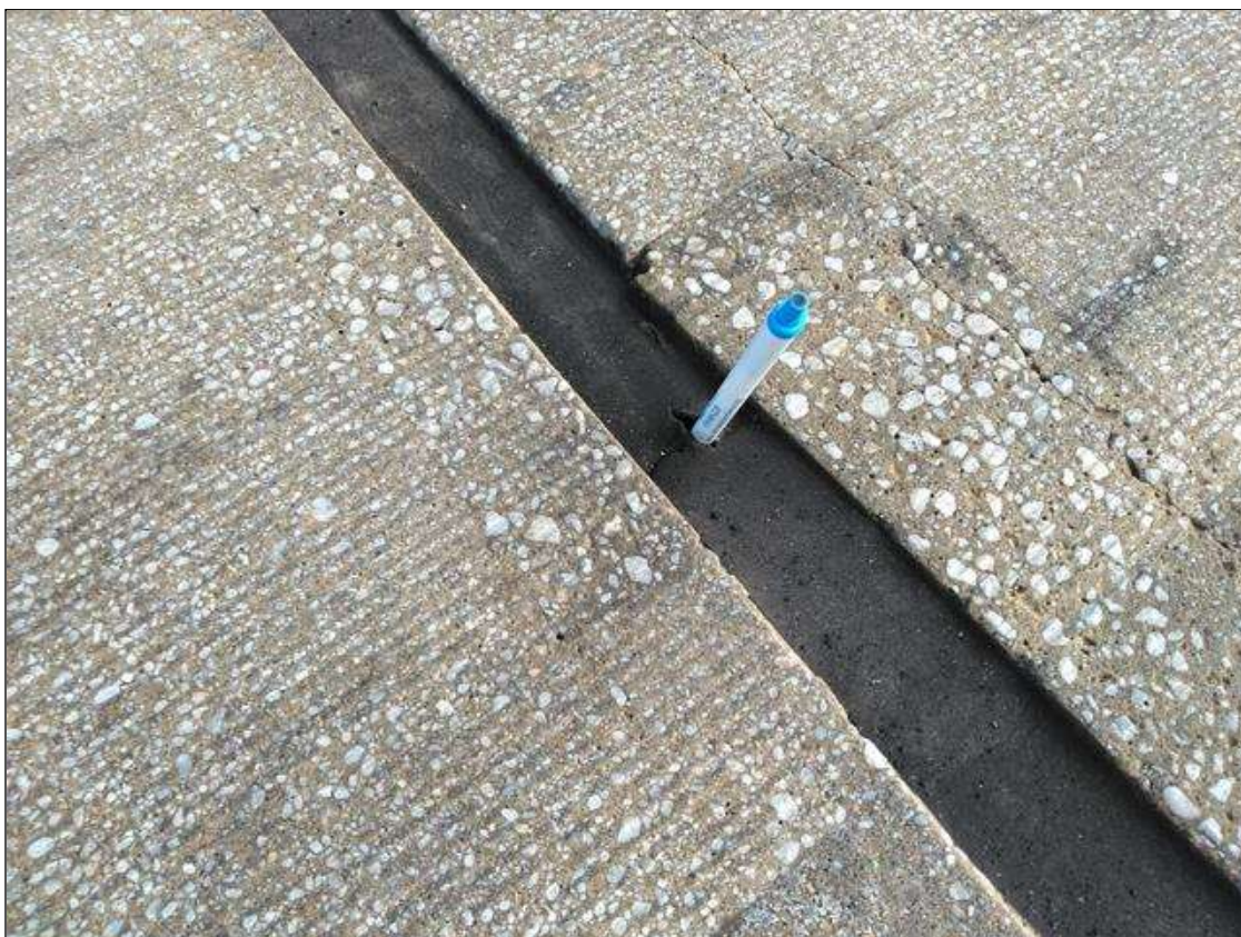
Span 203 Expansion Joint Bent 202: BENT 202, SCATTERED PARTIAL DEPTH CRACKING
