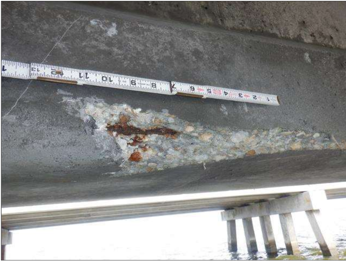
Span 59 Beam 1: (PAR) SOUTH FACE OF BOTTOM FLANGE AT 12 FEET FROM BENT 58, UNSOUND PATCHED AREA (30 INCHES X 12 INCHES) WITH SPALL (18 INCHES LONG X 7 INCHES HIGH X 2 INCHES DEEP) WITH EXPOSED RUSTED STRANDS (20 PERCENT SECTION LOSS)
