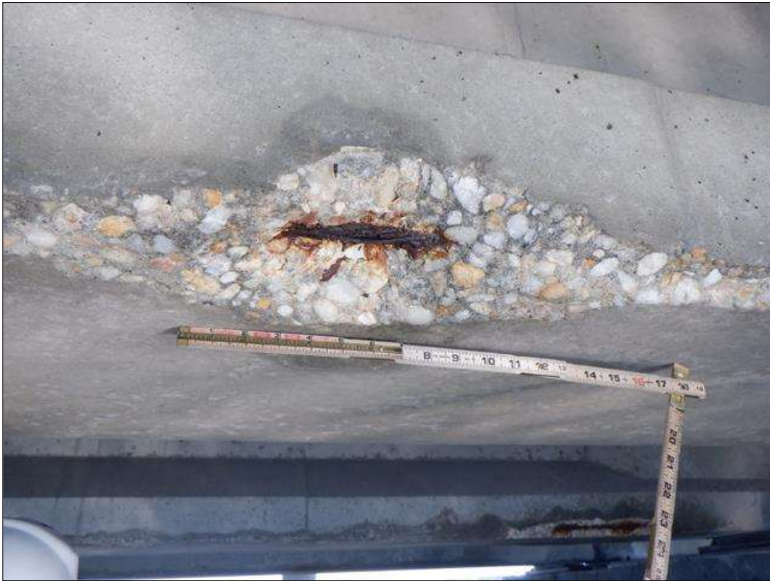
Span 216 Beam 3: (PAR) SOUTH FACE OF BOTTOM FLANGE, AT 9 FEET FROM BENT 216, SPALL (24 INCHES X 6 INCHES X 2 INCHES) WITH EXPOSED STRAND (30 PERCENT SECTION LOSS) ON STRAND
