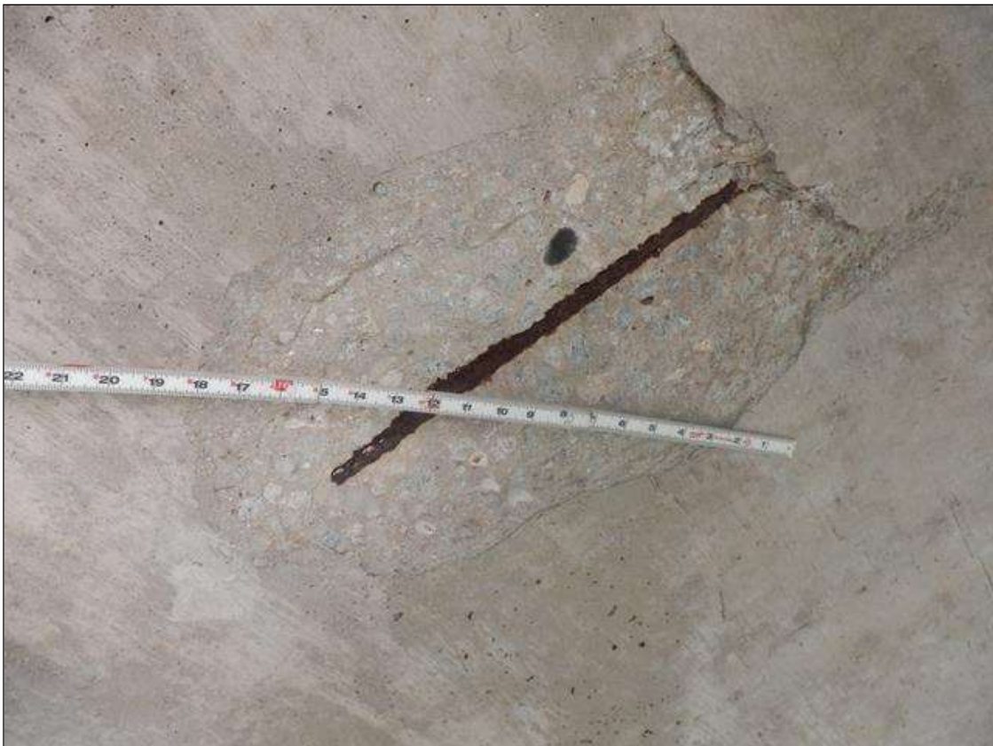
Span 182 Deck: UNDERSIDE OF DECK BAY 2 AT 13 FEET FROM BENT 181, MULTIPLE DELAMINATION/SPALL (18 INCHES DIAMETER X 1 INCH DEEP) WITH EXPOSED RUSTED REINFORCING (NO SECTION LOSS)
