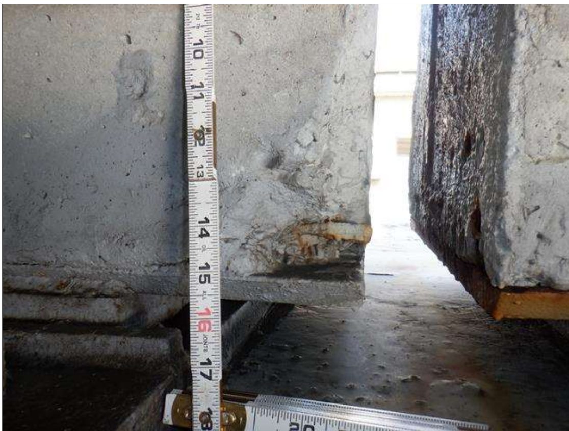
Span 78 Beam 1: SOUTH FACE OF BOTTOM FLANGE, AT BENT 78, SPALL (3 INCHES X 3 INCHES X 3 INCHES) WITH EXPOSED STRANDS (NO SECTION LOSS)
