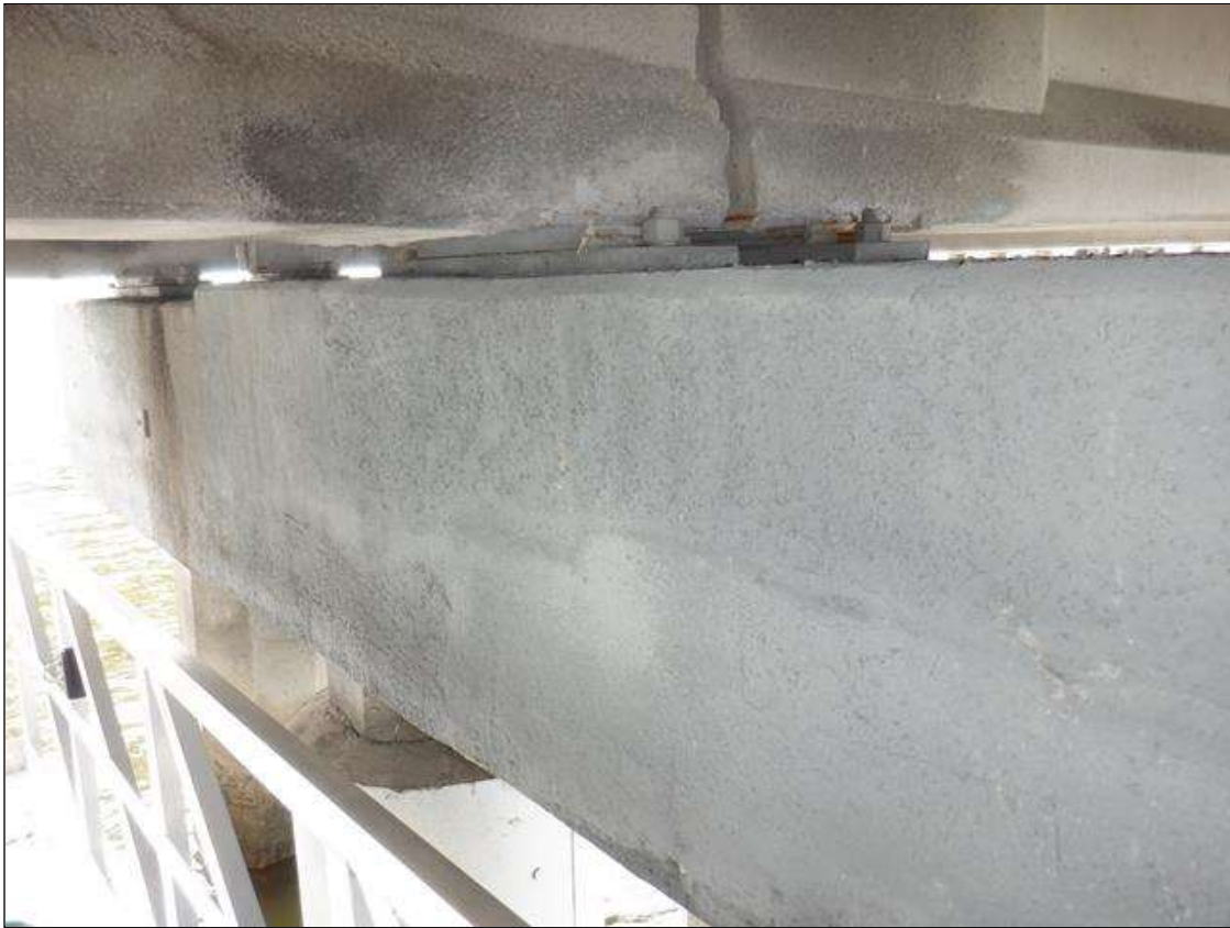
Bent 15 Cap 1: 5 FEET LONG X 1 FEET HIGH DELAMINATION ON TOP CAP STARTING AT BEAM 2
