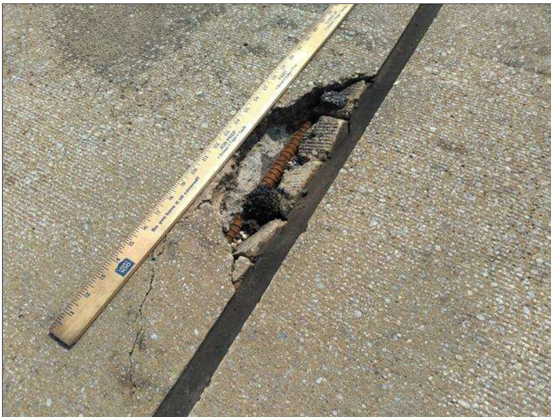
Span 156 Expansion Joint Bent 155: (PAR) LEFT LANE NEAR INCHES LEFT WHEEL PATH, SPALL (17INCHES X 5INCHES X 4 INCHES) WITH EXPOSED RUSTED REBAR
