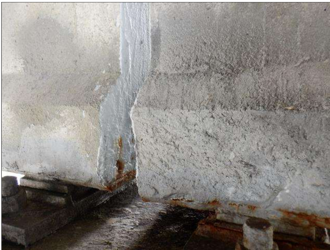
Span 69 Beam 1: SOUTH FACE OF BOTTOM FLANGE, AT BENT 68, SOUND PATCH (3 INCHES X 8 INCHES)
