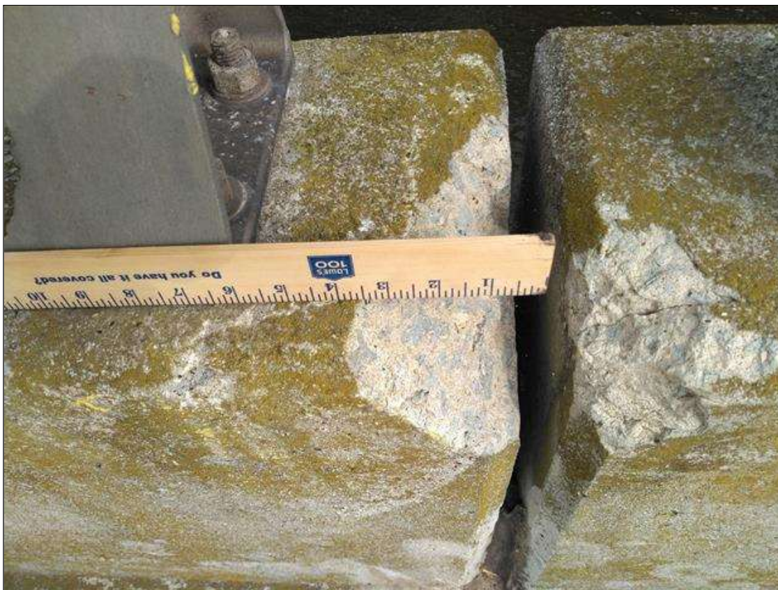
Span 5 Left Bridge Rail: AT BENT 5, SPALL (4INCHES X 10INCHES X 1INCH)
