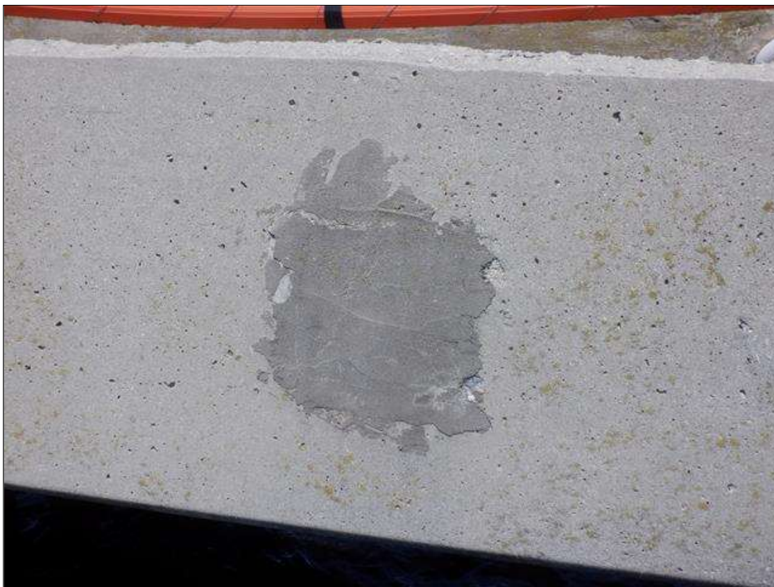
GROUT POCKET, SPAN 154
