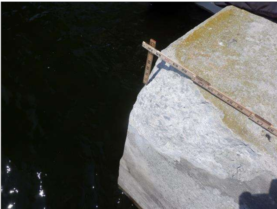
Bent 177 Footing: TOP SOUTHWEST CORNER, SPALL (32INCHES X 26INCHES X UP TO 4 INCHES)
