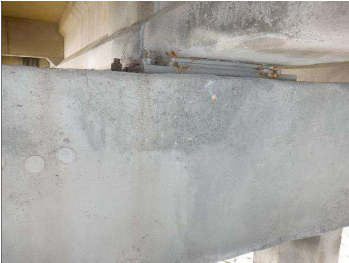
Bent 14 Cap 1: 6 INCHES X 6 INCHES DELAMINATION INCHES TOP EAST FACE CAP NEAR BEAM 2 , DID NOT FIND 9/12/22
