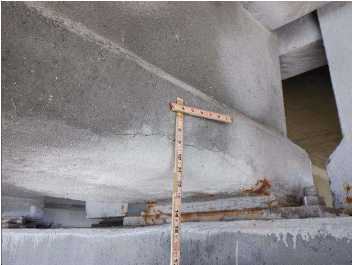
Span 152 Beam 3: 13 INCHES LONG X 1/16 INCH WIDE CRACK AT END OF BEAM, AT BENT 152
