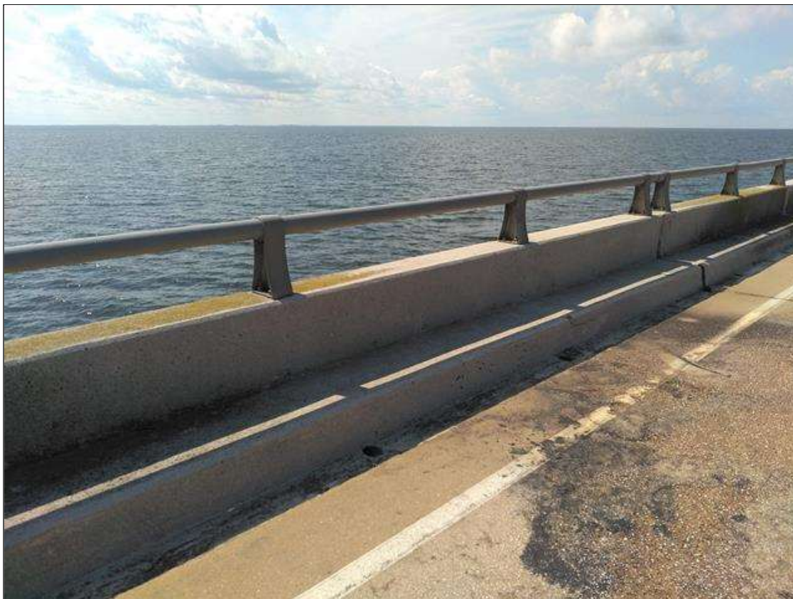
Span 148 Right Bridge Rail: FIRST 14 FEET OF RAIL APPEARS REPAIRED FROM IMPACT
