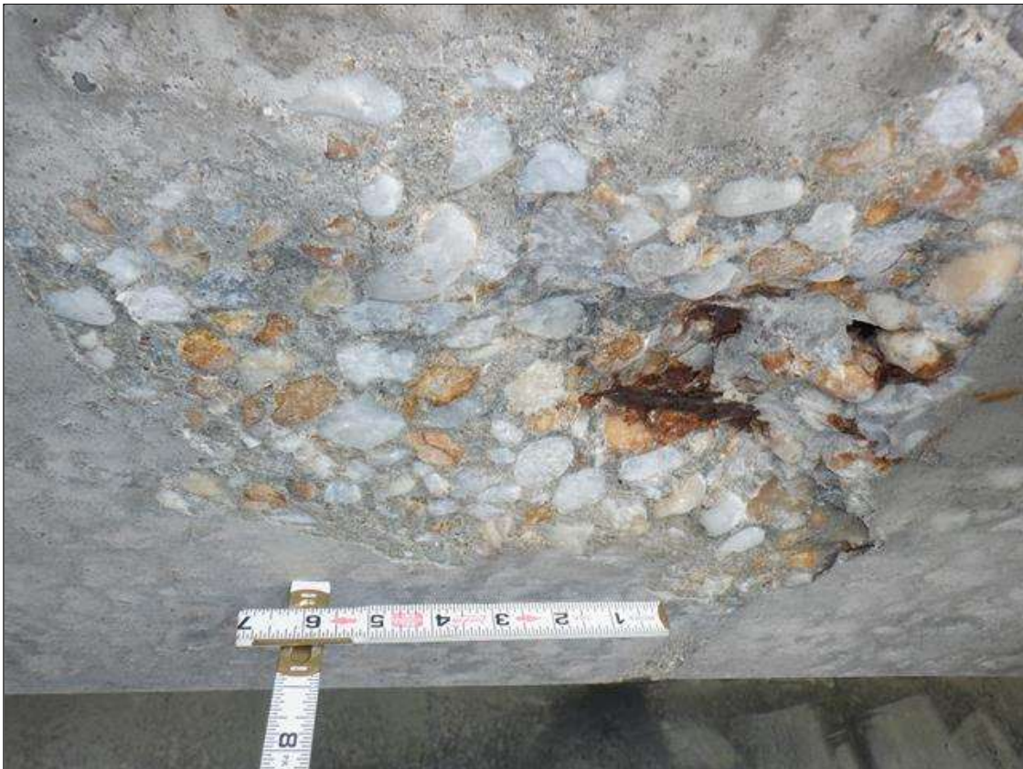
Span 160 Beam 2: (PAR) BOTTOM OF BOTTOM FLANGE 22 FEET FROM BENT 159, SPALL (10 INCH DIAMETER X UP TO 1 INCH DEEP) WITH EXPOSED RUSTED STRANDS (10 PERCENT SECTION LOSS)
