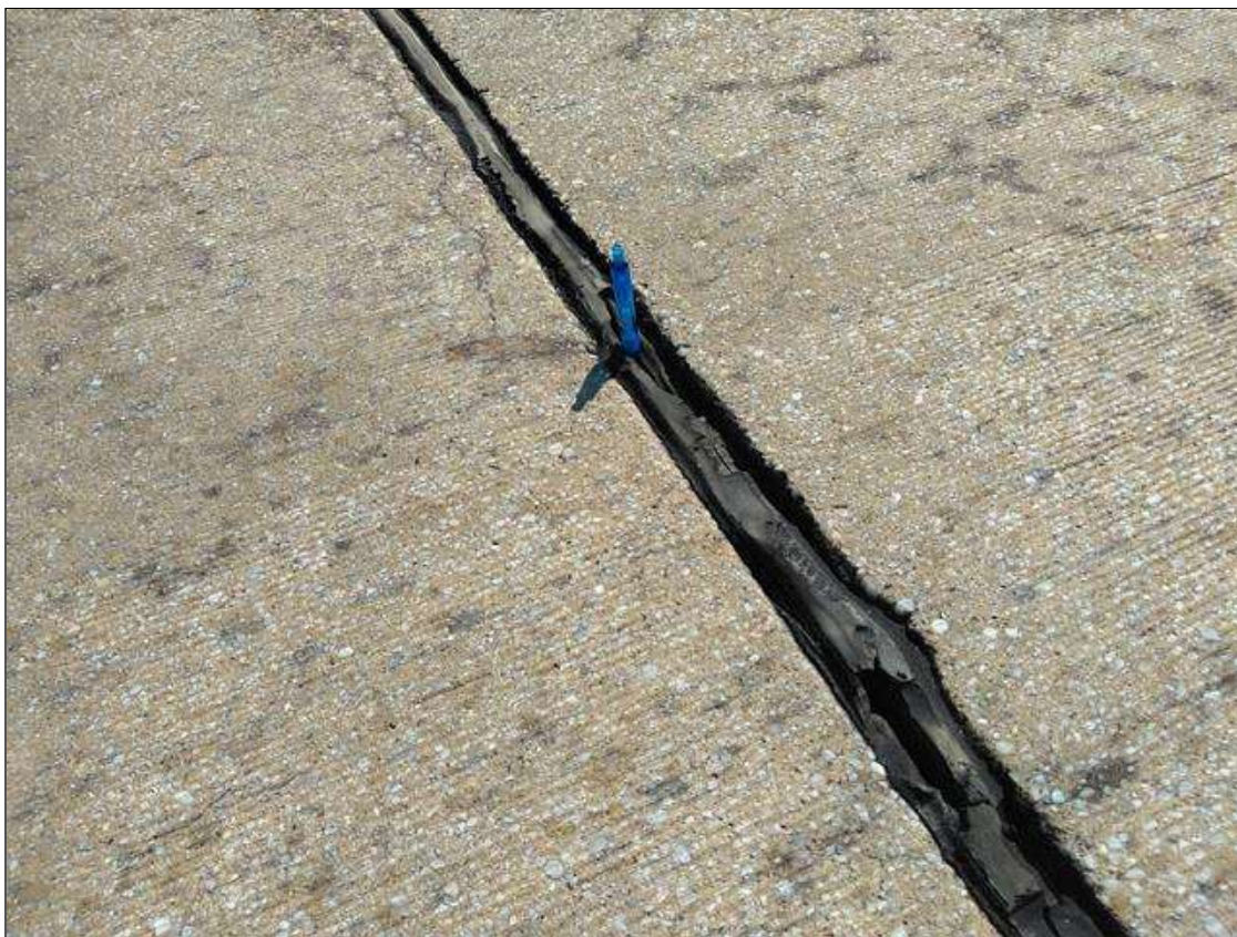
Span 189 Expansion Joint Bent 188: BENT 188, FULL DEPTH X FULL WIDTH TORN JOINT
