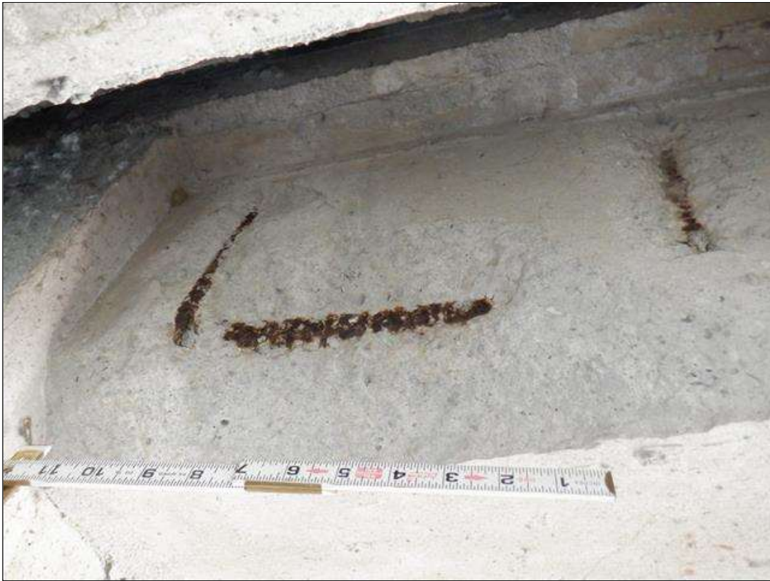
Span 32 Beam 1: END DIAPHRAGM OVER BENT 31, SPALL (11 INCHES HIGH X 30 INCHES WIDE X 2 INCHES DEEP) WITH (4) FOUR EXPOSED RUSTED REINFORCING (NO LOSS)
