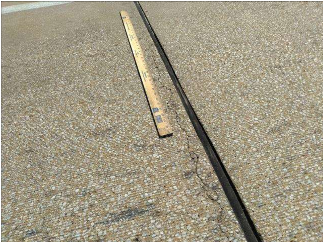
Span 180 Expansion Joint Bent 179: AT BENT 179, THROUGHOUT RIGHT LANE, EDGE DELAMINATIONS
