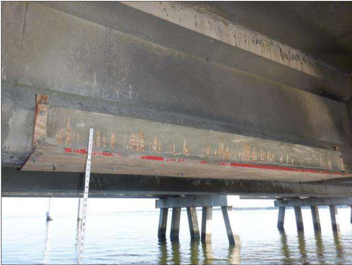
Span 155 Beam 2: 8 FEET LONG X FULL WIDTH SOUND PATCHED AREA ON BOTTOM FLANGE, SOUTH AND BOTTOM FACES, 10 FEET FROM BENT 154 WITH FORMWORK IN PLACE
