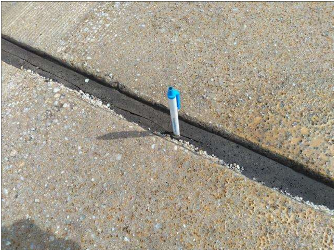
Span 246 Expansion Joint Bent 245: AT BENT 245, INTERMITTENT PARTIAL DEPTH CRACKING THROUGHOUT RIGHT LANE AND LEFT SHOULDER
