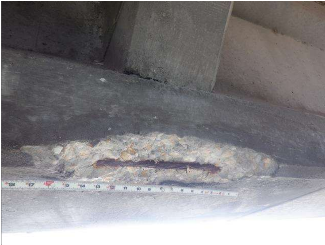
Span 174 Beam 4: (PAR) NORTH FACE OF BOTTOM FLANGE AT 20 FEET FROM BENT 173, SPALL (18 INCHES X 4 1/2 INCHES X 2 1/2 INCHES) WITH TWO (2) EXPOSED STRANDS (20 PERCENT SECTION LOSS) ON STRAND
