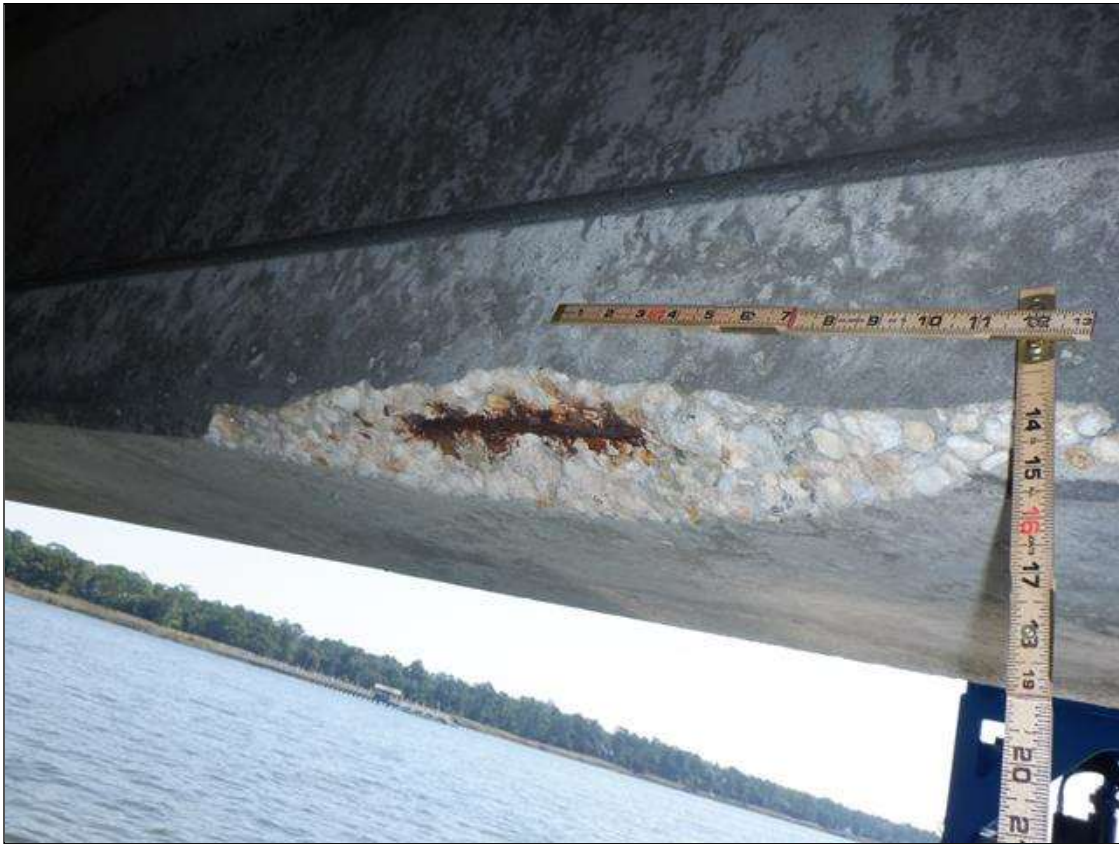
Span 229 Beam 4: (PAR) BOTTOM FLANGE NORTH FACE AT 5 FEET FROM BENT 228, SPALL (32 INCHES LONG X 3 INCHES HIGH X 5 INCHES WIDE X UP TO 1.5 INCHES DEEP) WITH EXPOSED RUSTED STRAND (20 PERCENT SECTION LOSS)
