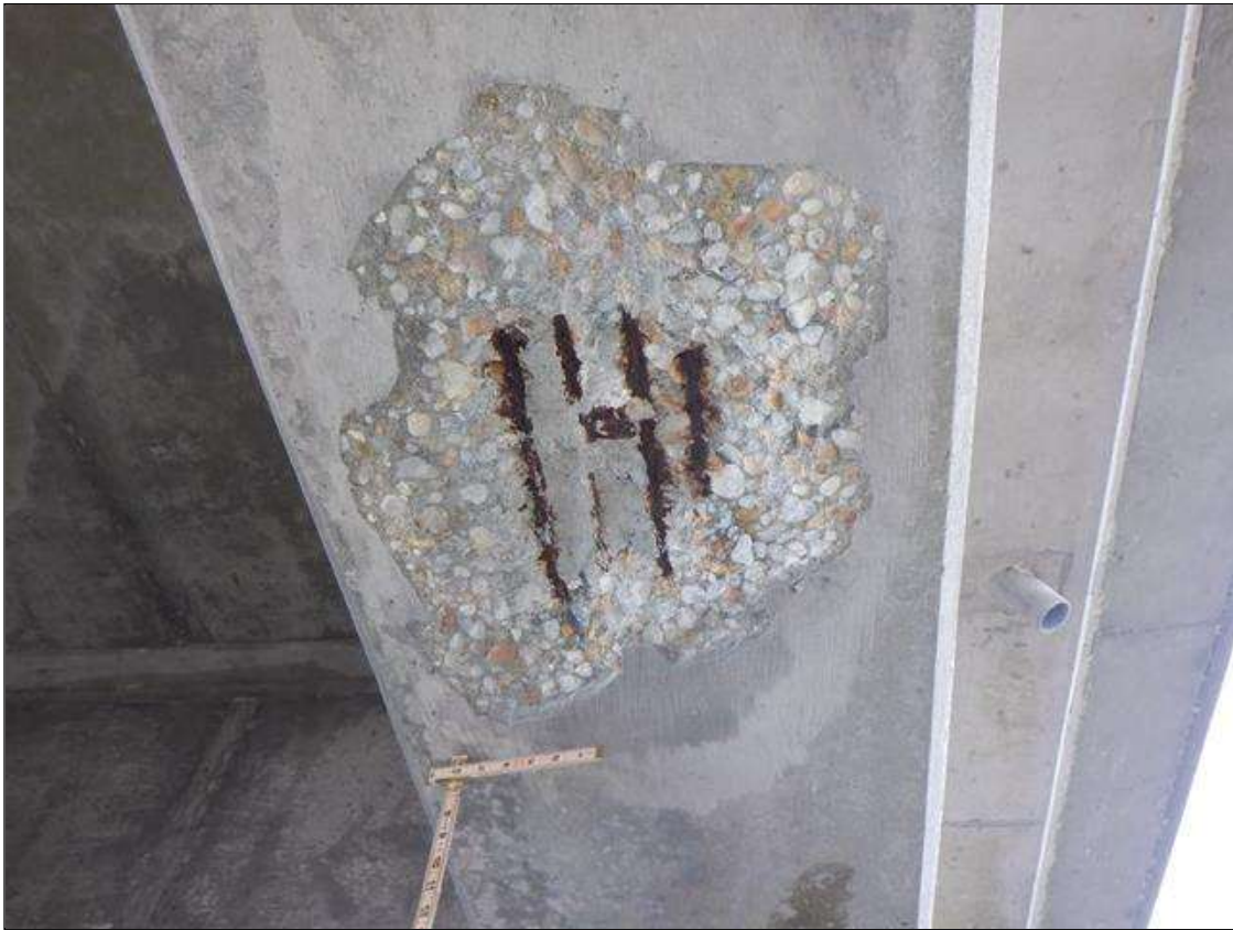
Span 142 Beam 1: (PAR) BOTTOM OF BOTTOM FLANGE AT MIDSPAN, SPALL (24 INCHES LONG X 16 INCHES WIDE X 1.5 INCHES DEEP) WITH (4) FOUR EXPOSED RUSTED STRANDS (20 PERCENT SECTION LOSS)
