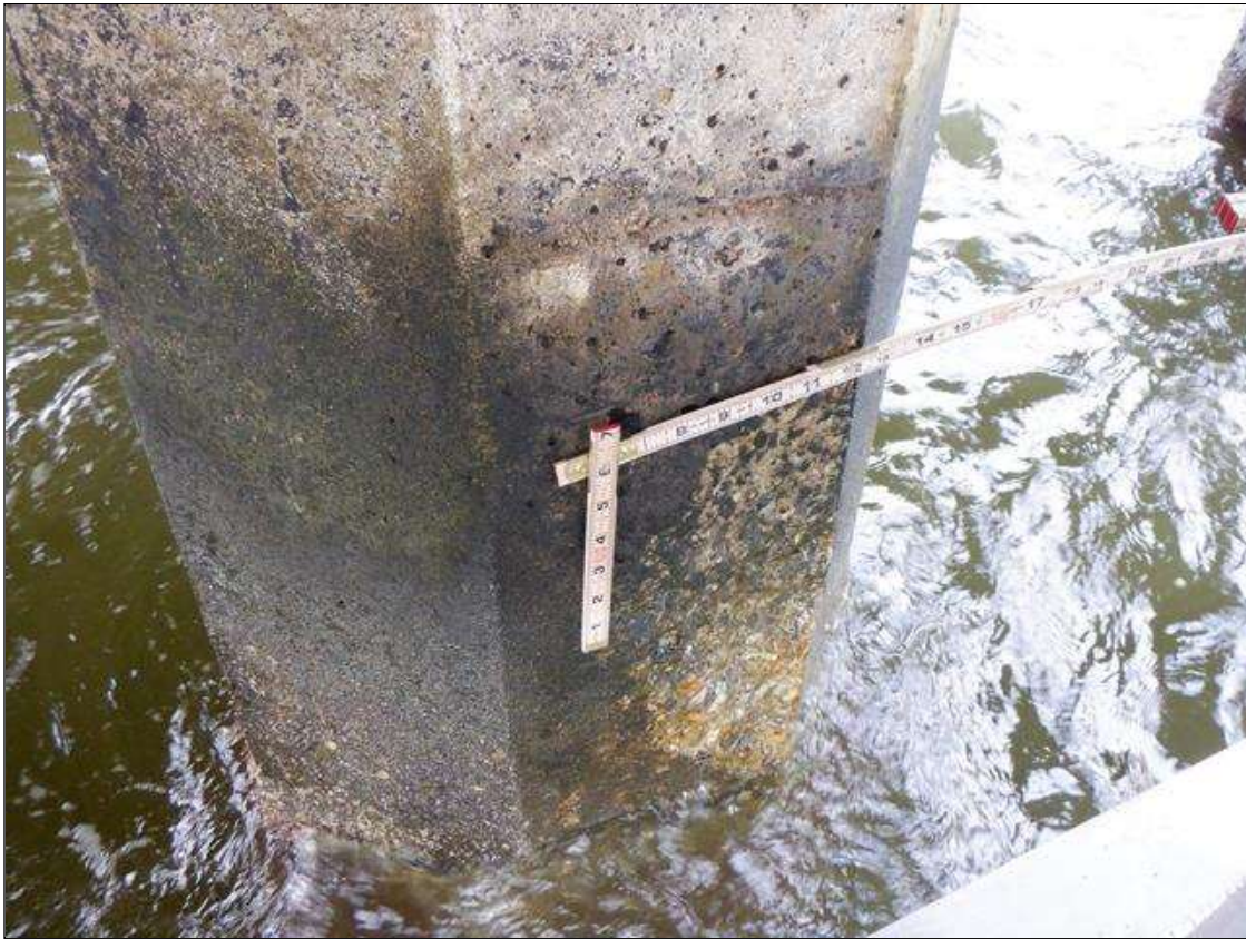
Bent 140 Pile 3: EAST FACE NEAR WATERLINE, SPALL (18 INCHES X 8 INCHES X 1 INCHES)
