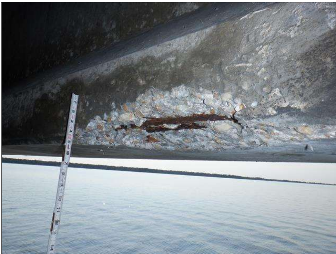
Span 155 Beam 5: (PAR) BOTTOM FLANGE NORTH FACE AT 25 FEET FROM BENT 154, SPALL (24 INCHES LONG X 4 INCHES HIGH X 2 INCHES DEEP) WITH (2) TWO EXPOSED RUSTED STRANDS (30 PERCENT SECTION LOSS)
