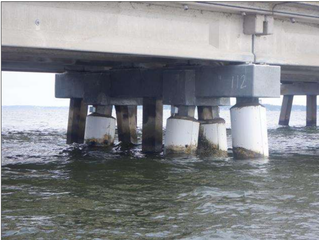
TYPICAL INTERIOR BENT PROFILE, SEVEN PILES IN VIEW
