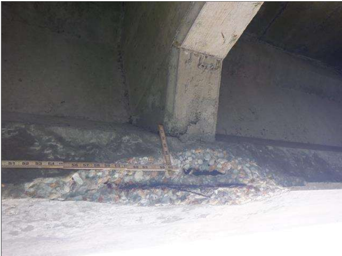
Span 116 Beam 4: (PAR) NORTH FACE OF BOTTOM FLANGE AT 20 FEET FROM BENT 115, SPALL (24 INCHES X 6 INCHES X 4 INCHES) WITH BROKEN STRANDS (100 PERCENT SECTION LOSS) ON STRAND
