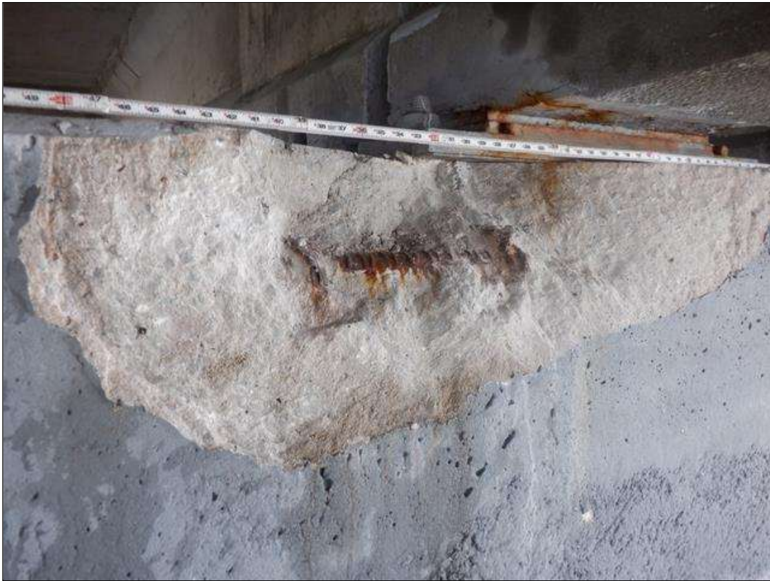
Bent 199 Cap 1: (PAR) WEST FACE BELOW BEAM 2, SPALL (4 FEET X 1 FOOT X UP TO 8 INCHES DEEP) WITH ONE (1) EXPOSED PRIMARY REBAR (NO SECTION LOSS), UNDERMINING OF BEARING (8 INCHES X 2 INCHES AVERAGE)
