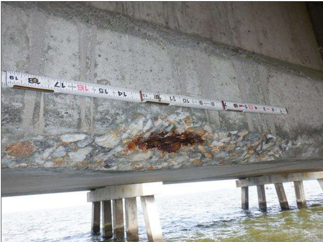
Span 67 Beam 1: (PAR) BOTTOM FLANGE SOUTH FACE AT 20 FEET FROM BENT 67, SPALL (18 INCHES LONG X 3 INCHES HIGH X UP TO 2 INCHES DEEP) WITH EXPOSED RUSTED STRANDS (10 PERCENT SECTION LOSS)
