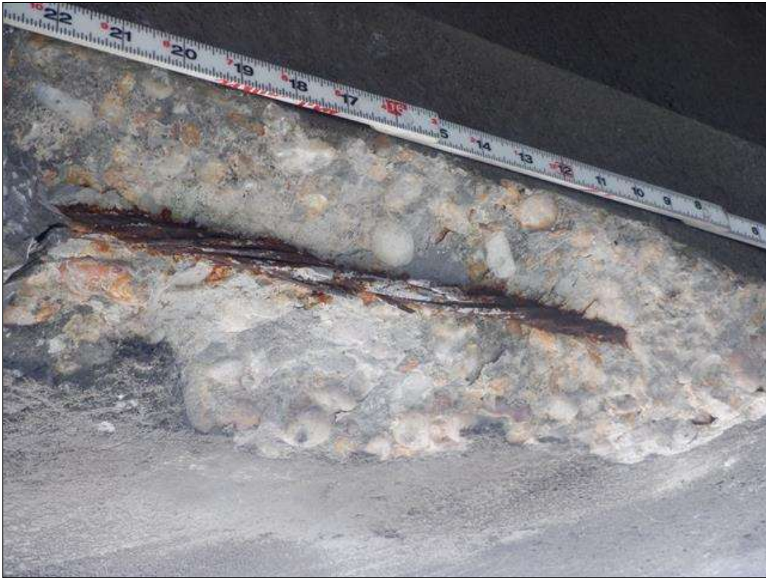
Span 187 Beam 4: (PAR) NORTH FACE OF BOTTOM FLANGE AT 2 FEET FROM BENT 186, SPALL (2 FEET X 6 INCHES X 2 INCHES DEEP) WITH ONE (1) EXPOSED AND PARTIALLY SEVERED STRAND
