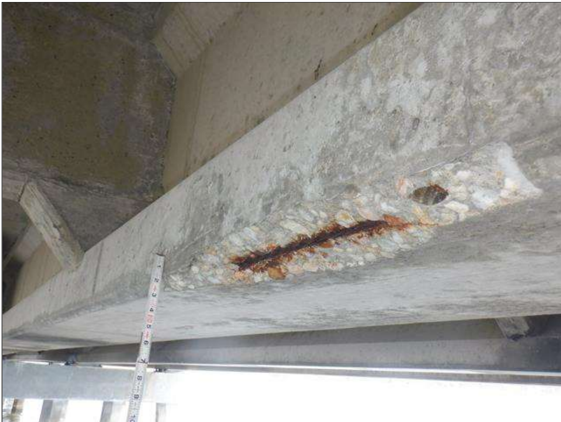
Span 212 Beam 2: (PAR) NORTH FACE OF BOTTOM FLANGE AT 15 FEET FROM BENT 211, SPALL (24 INCHES X 5 INCHES X 1.5 INCHES) WITH EXPOSED RUSTED STRANDS (10 PERCENT SECTION LOSS) ON STRANDS
