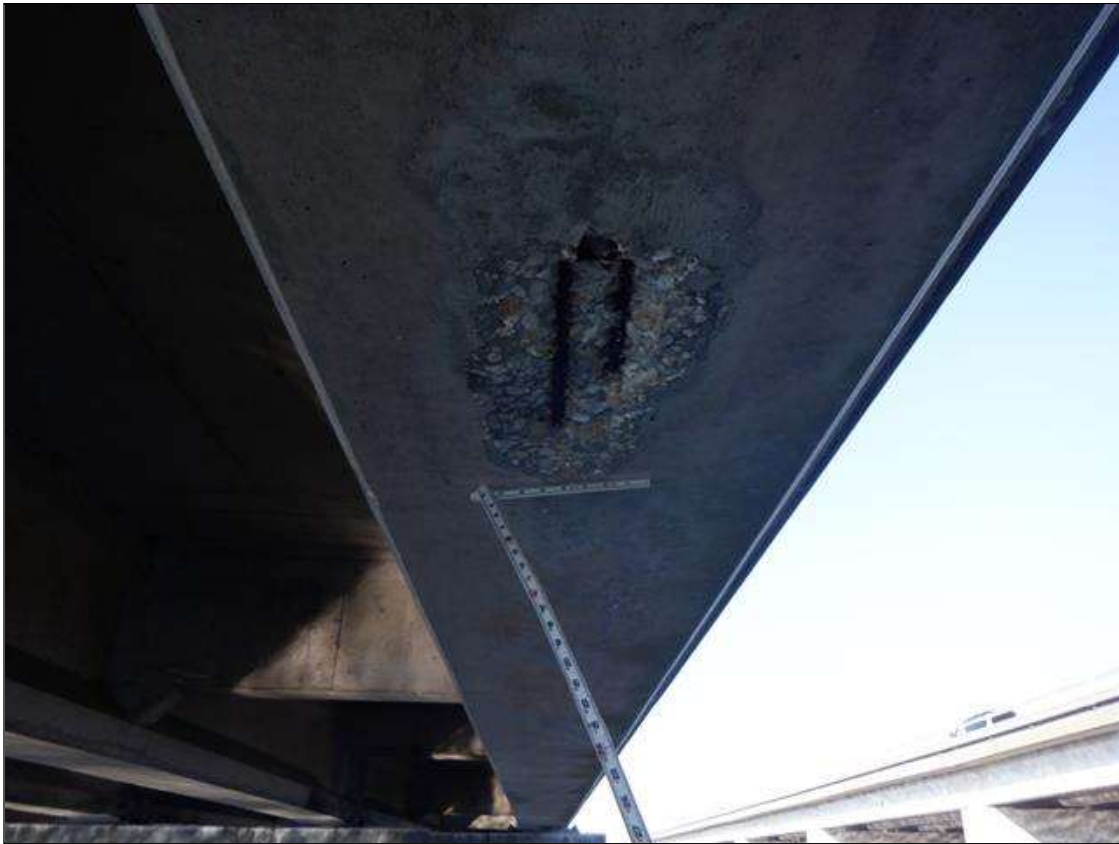
Span 237 Beam 1: (PAR) UNDERSIDE OF BOTTOM FLANGE, AT 24 FEET FROM BENT 237, SPALL (18 INCHES X 8 INCHES X 1 IN) WITH (2) EXPOSED RUSTED STRANDS (10 PERCENT SECTION LOSS) ON STRAND
