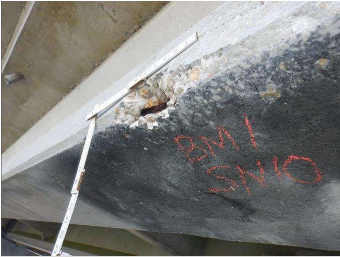
Span 10 Beam 1: (PAR) SOUTH FACE OF BOTTOM FLANGE AND WEB AT 7 FEET FROM BENT 9, PATCHED AREA (48 INCHES X 18 INCHES), WITH SPALL (10 INCHES X 3 INCHES X UP TO 2 INCHES DEEP) WITH EXPOSED RUSTED STRANDS (UP TO 50 PERCENT SECTION LOSS)
