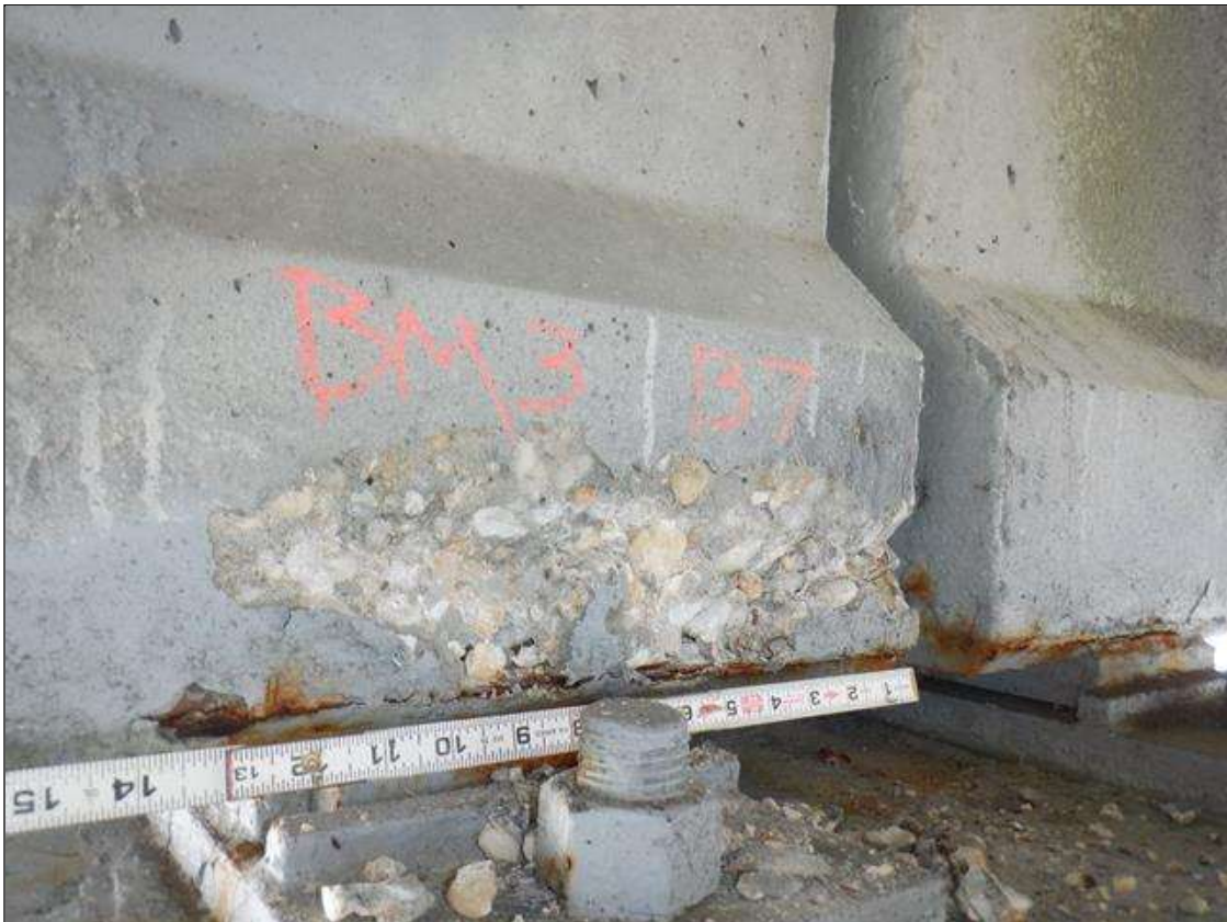
Span 8 Beam 3: NORTH FACE BOTTOM FLANGE AT BENT 7, SPALL (13 INCHES LONG X 5 INCHES HIGH X UP TO 1 INCH DEEP)
