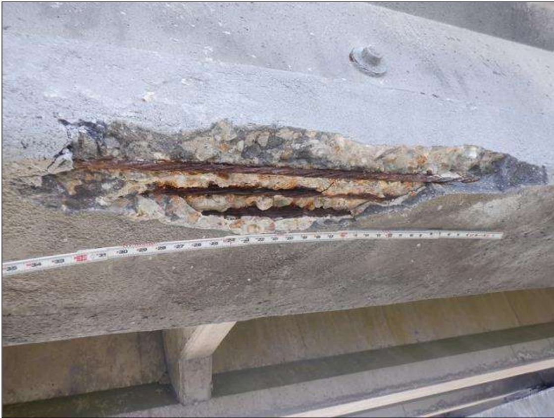
Span 171 Beam 1: (PAR) NORTH FACE AND UNDERSIDE, SPALL (2 1/2 INCHES X 6 INCHES X UP TO 2 INCHES DEEP) WITH FOUR EXPOSED STARNDs (50 PERCENT LOSS)
