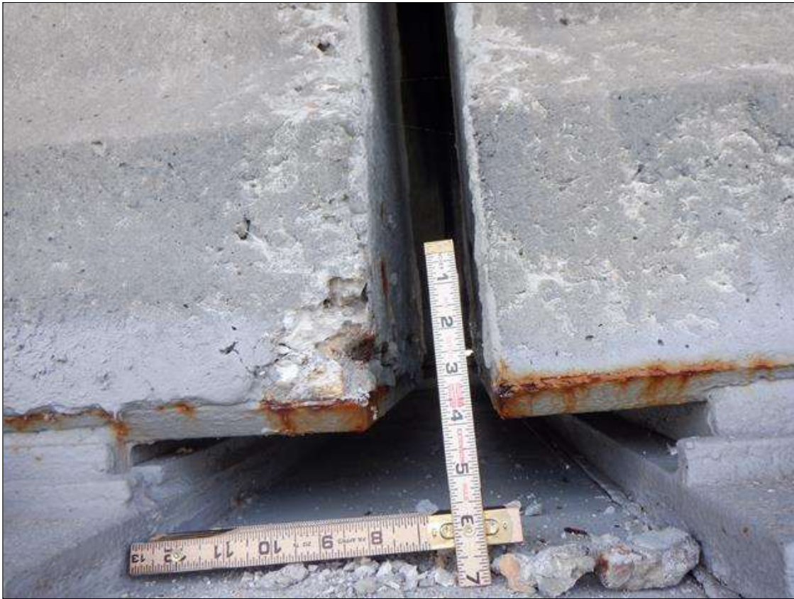
Span 103 Beam 1: (PAR) SOUTH FACE OF BOTTOM FLANGE AT BENT 103, SPALL (3 INCHES LONG X 3 INCHES HIGH X 2 INCHES DEEP WITH (1) EXPOSED STRAND (NO LOSS)
