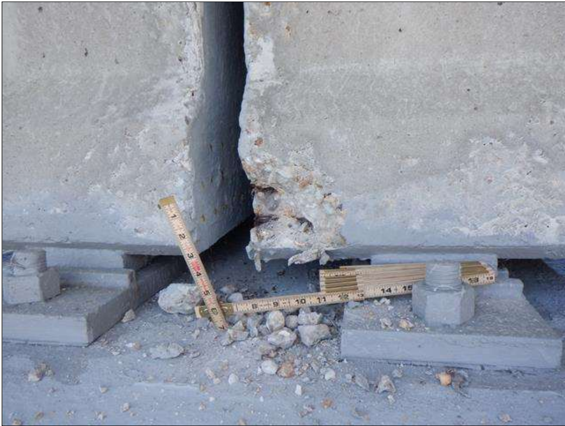
Span 110 Beam 4: (PAR) SOUTH FACE OF BOTTOM FLANGE AT BENT 109, SPALL (5 INCHES LONG X 5 INCHES HIGH X 2 INCHES DEEP) WITH (1) EXPOSED STRAND (NO LOSS)
