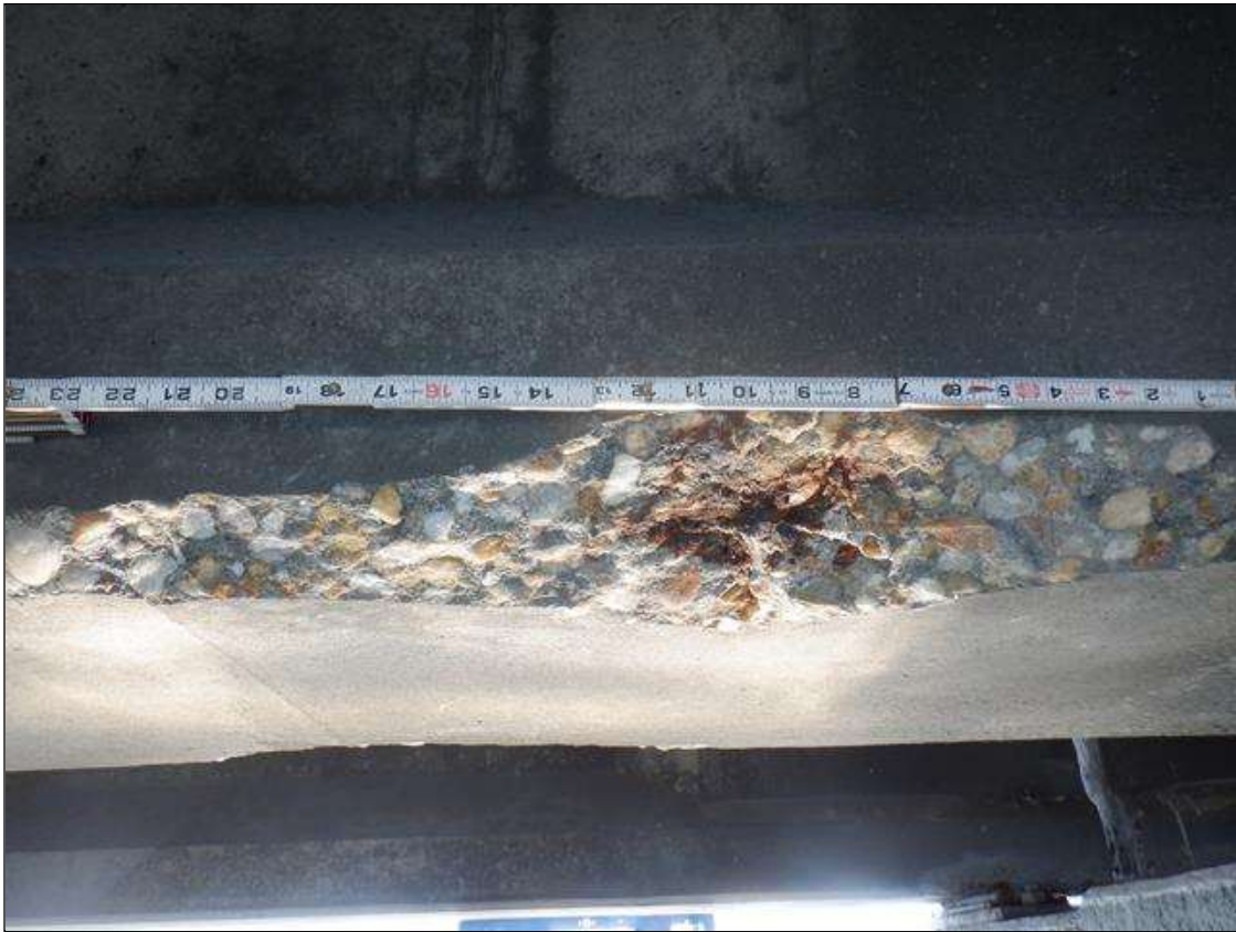
Span 162 Beam 3: (PAR) BOTTOM FLANGE BOTH FACES 5 FEET FROM BENT 161, (2) TWO SPALLS (28 INCHES LONG X 5 INCHES WIDE X 1.5 INCHES DEEP) WITH EXPOSED RUSTED STRANDS (10 PERCENT SECTION LOSS)
