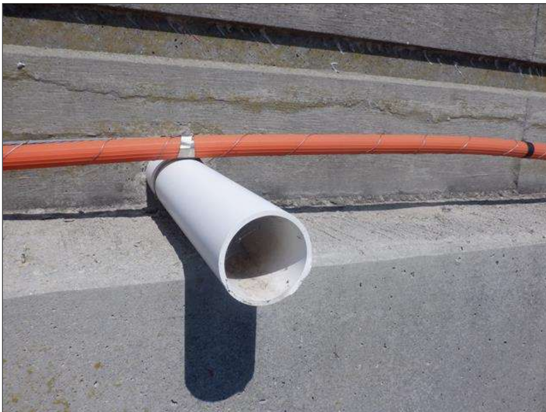
TYPICAL DECK DRAIN, SPAN 154
