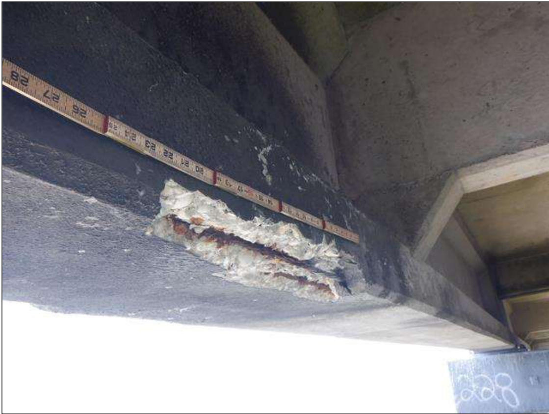
Span 229 Beam 4: (PAR) BOTH FACES OF BOTTOM FLANGE AT 21 FEET FROM BENT 228, FAILED PATCH/SPALL (26 INCHES LONG X 3 INCHES HIGH X 6 INCHES WIDE X UP TO 2.5 INCHES DEEP) WITH (2) TWO EXPOSED RUSTED STRANDS WITH (1) ONE PARTIALLY SEVERED STRAND
