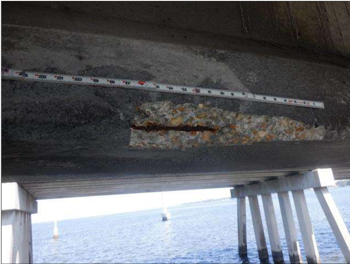
Span 192 Beam 1: (PAR) SOUTH FACE OF BOTTOM FLANGE AT 8 FEET FROM BENT 191, PATCHED AREA (20 INCHES X 4 INCHES) WITH ASSOCIATED SPALL (16 INCHES X 4 INCHES X 2 INCHES DEEP) WITH ONE (1) EXPOSED STRAND (10 PERCENT LOSS)
