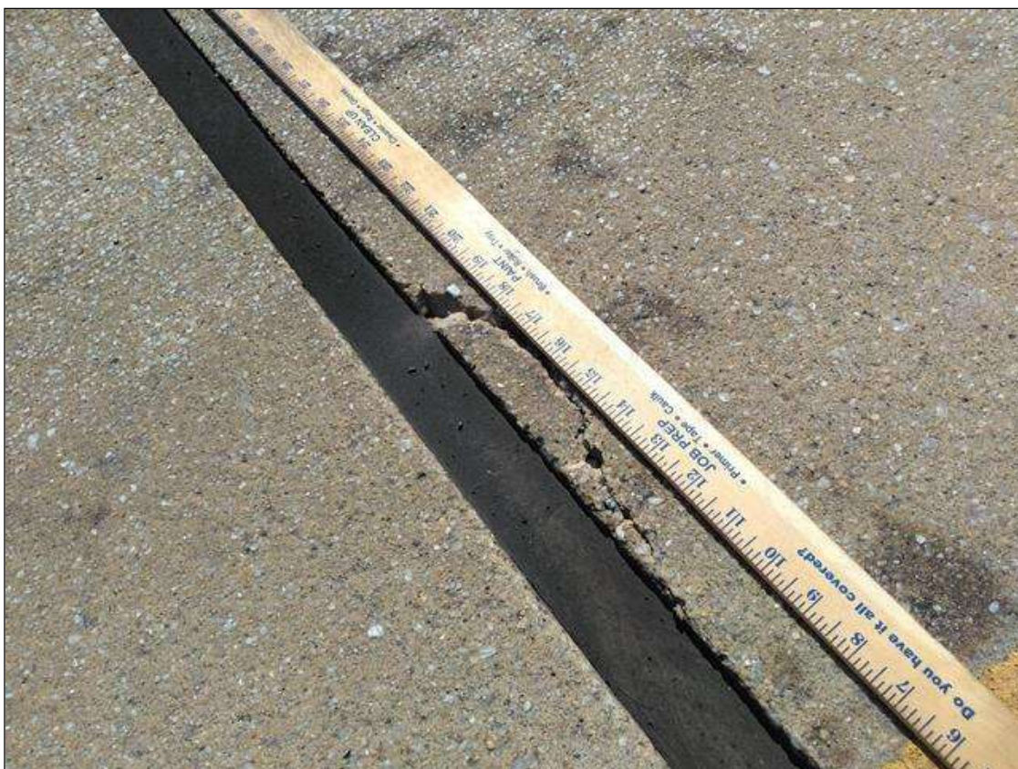
Span 178 Expansion Joint Bent 177: AT BENT 177, LEFT LANE DELAMINATION 8 INCH WIDE X 2 INCH LONG
