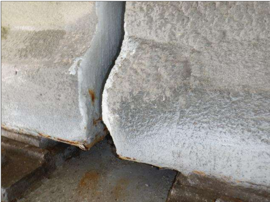
Span 69 Beam 3: SOUTH FACE OF BOTTOM FLANGE, AT BENT 68, SOUND PATCH (8 INCHES X 10 INCHES)
