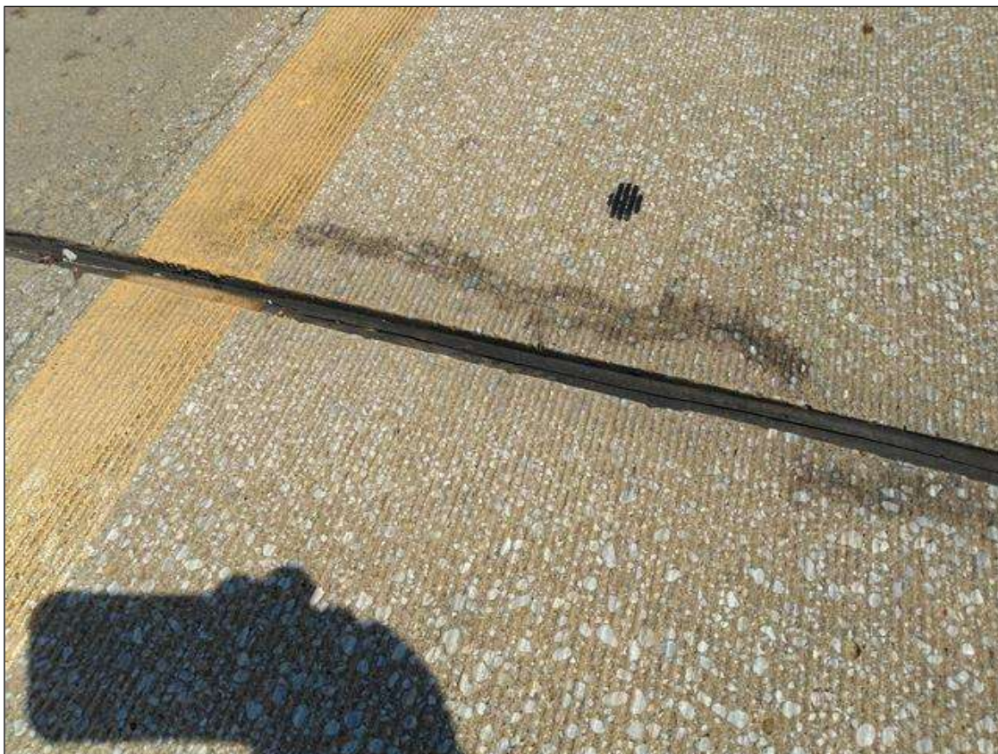
Span 56 Expansion Joint Bent 55: LEFT LANE NEAR CURB, DELAMINATION (2FEET X 3 INCHES)
