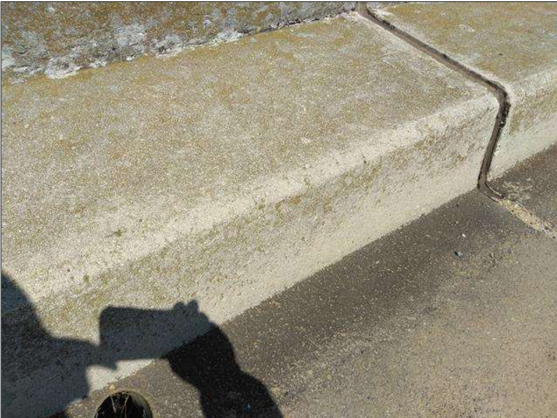
Span 51 Left Bridge Rail: SCATTERED THROUGHOUT, (3) VERTICAL CRACKS (FULL HEIGHT X HAIRLINE) WITH EFFLORESCENCE (DEFECT NOT FOUND 9/12/22)
