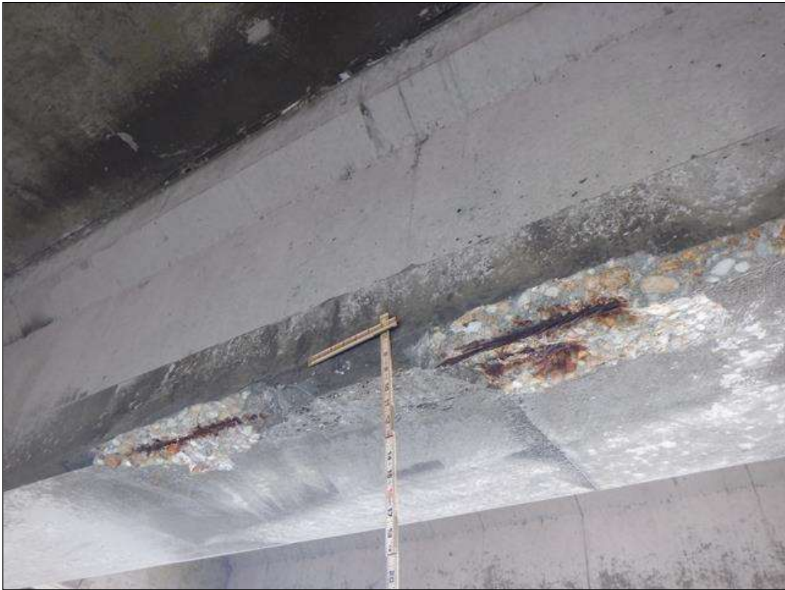
Span 133 Beam 3: (PAR) NORTH FACE OF BOTTOM FLANGE AT MIDSPAN, (2) TWO ADJACENT SPALLS (UP TO 24 INCHES X 6 INCHES X 2 INCHES) WITH BROKEN STRANDS (100 PERCENT SECTION LOSS) ON STRAND
