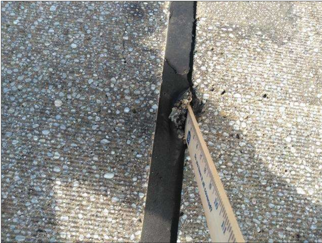
Span 19 Expansion Joint Bent 18: BENT 18 JOINT, LEFT LANE SPALL 3 INCH WIDE X 1 INCH LONG X 1 INCH DEEP, ADHESION FAILURE
