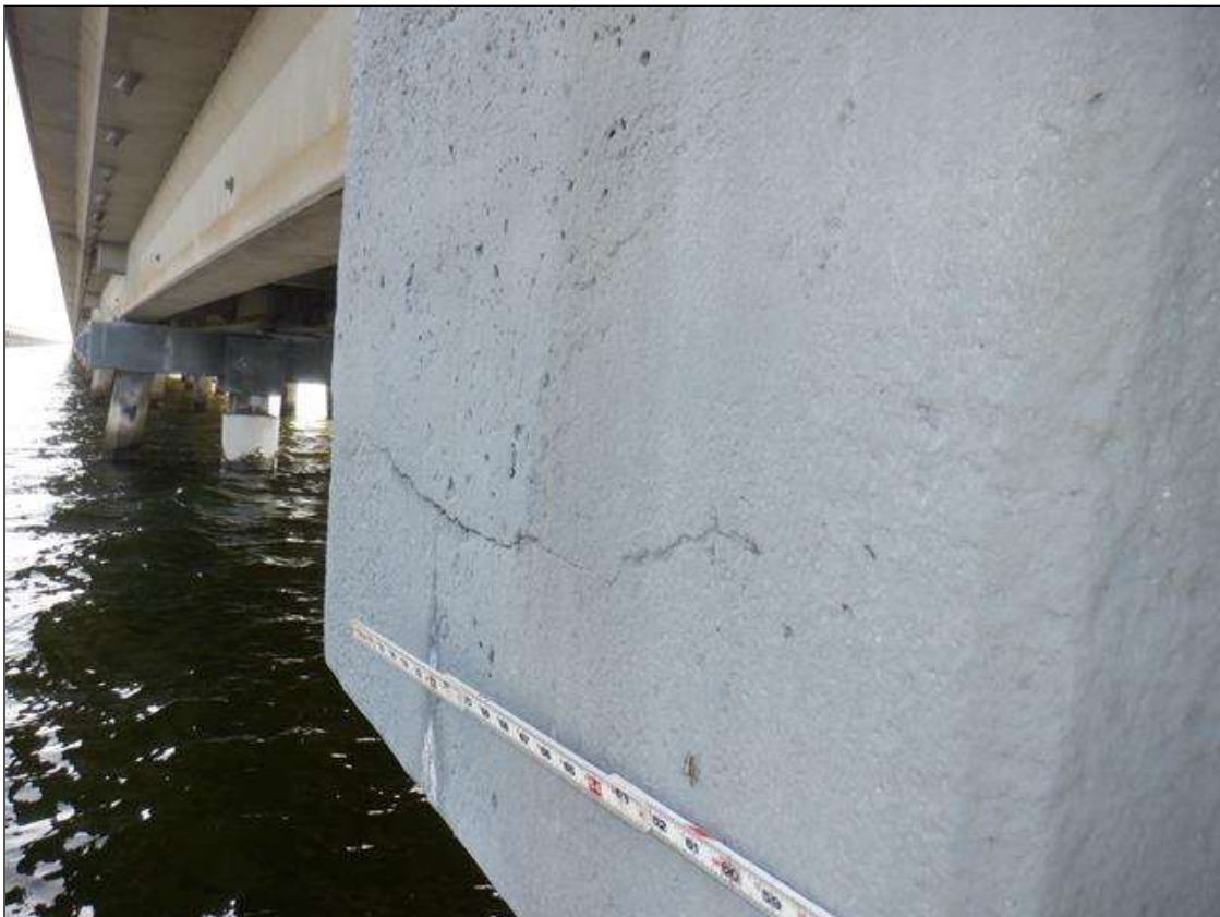
Bent 31 Cap 1: 1/16 INCHES HORIZONTAL CRACK 2 FEET LONG, 1/16 INCHES VERTICAL CRACK 9 INCHES LONG ON NORTH FACE OF CAP
