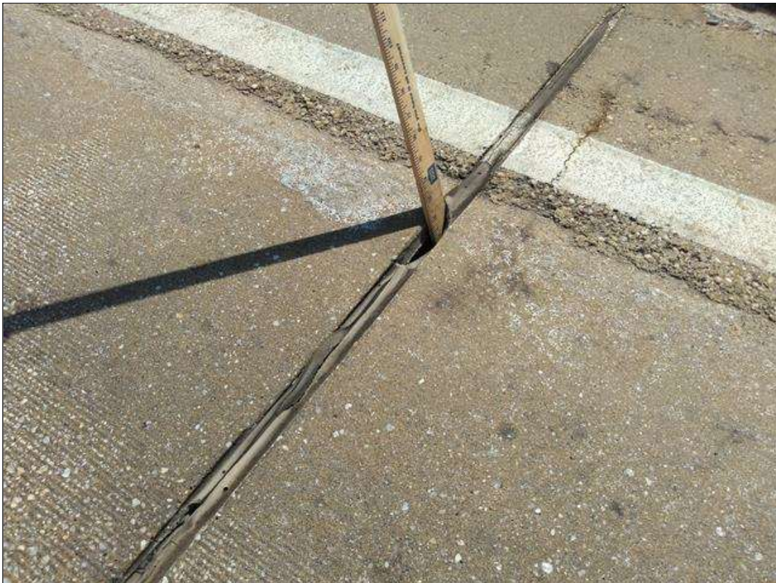
Span 50 Expansion Joint Bent 49: BOTH SHOULDERS, SEAL DAMAGE (2) 4 INCH LONG PIECES MISSING IN RIGHT SHOULDER
