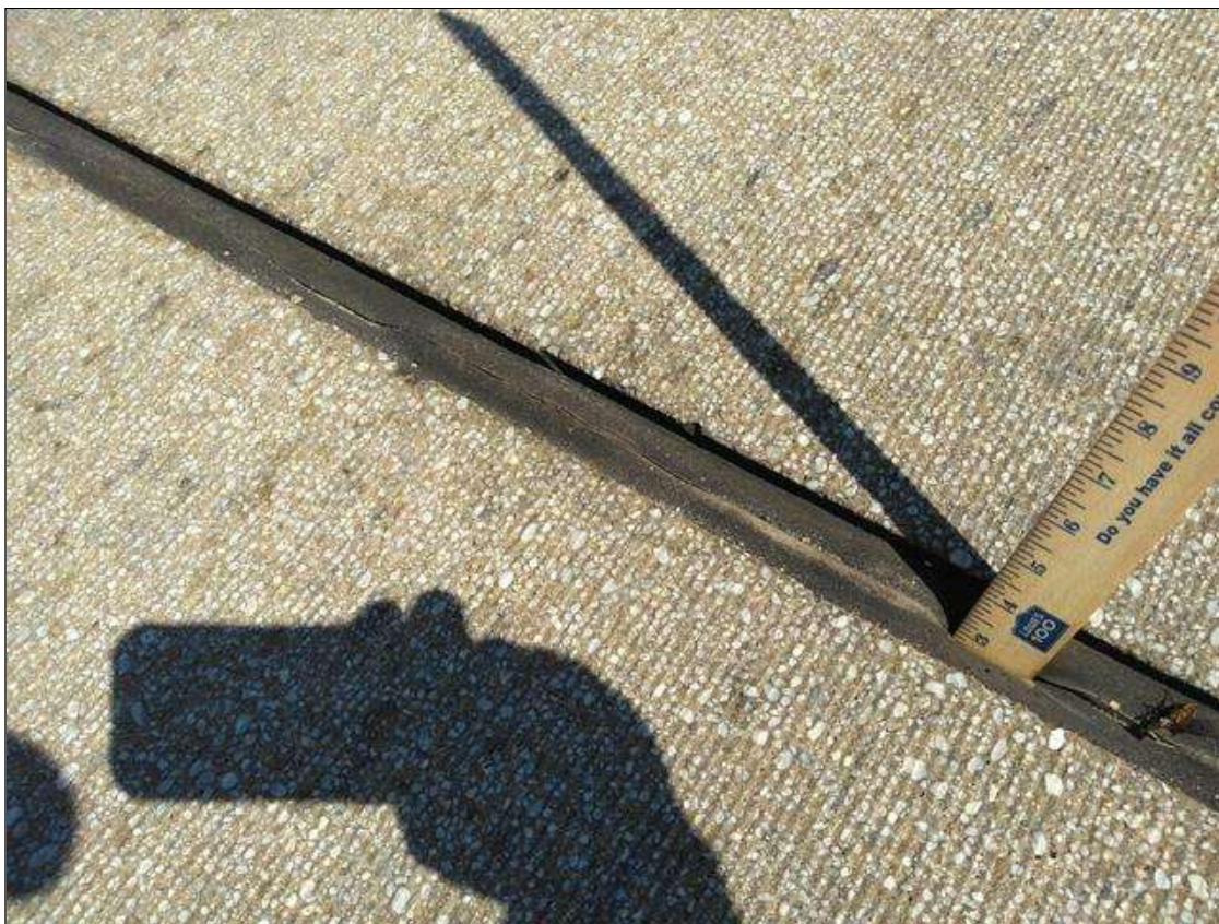
Span 38 Expansion Joint Bent 37: AT BENT 37, FULL DEPTH FULL WIDTH CRACK
