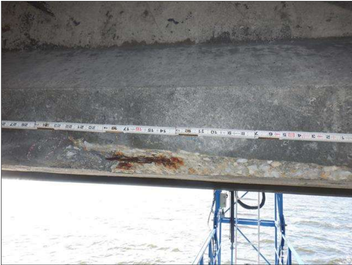
Span 54 Beam 3: (PAR) NORTH FACE OF BOTTOM FLANGE AT 15FEET FROM BENT 53, SPALL (UP TO 21 INCHES X 7 INCHES X 2 INCHES) WITH EXPOSED RUSTED STRAND, ADJACENT DELAMINATION (8INCHES DIAMETER) AND SECTION LOSS (10 PERCENT) ON STRAND
