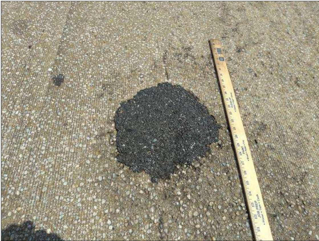
Span 60 Deck: RIGHT LANE 20 FEET FROM BENT 60, PATCHED AREA 12 INCH DIAMETER
