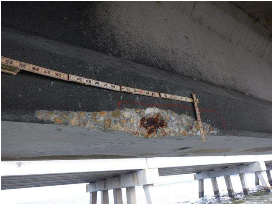
Span 138 Beam 1: SOUTH FACE OF BOTTOM FLANGE AT 22 FEET FROM BENT 137, SPALL (27 INCHES LONG X 3 INCHES HIGH X 4 INCHES WIDE X 1.5 INCHES DEEP) WITH EXPOSED RUSTED REINFORCING (NO LOSS)
