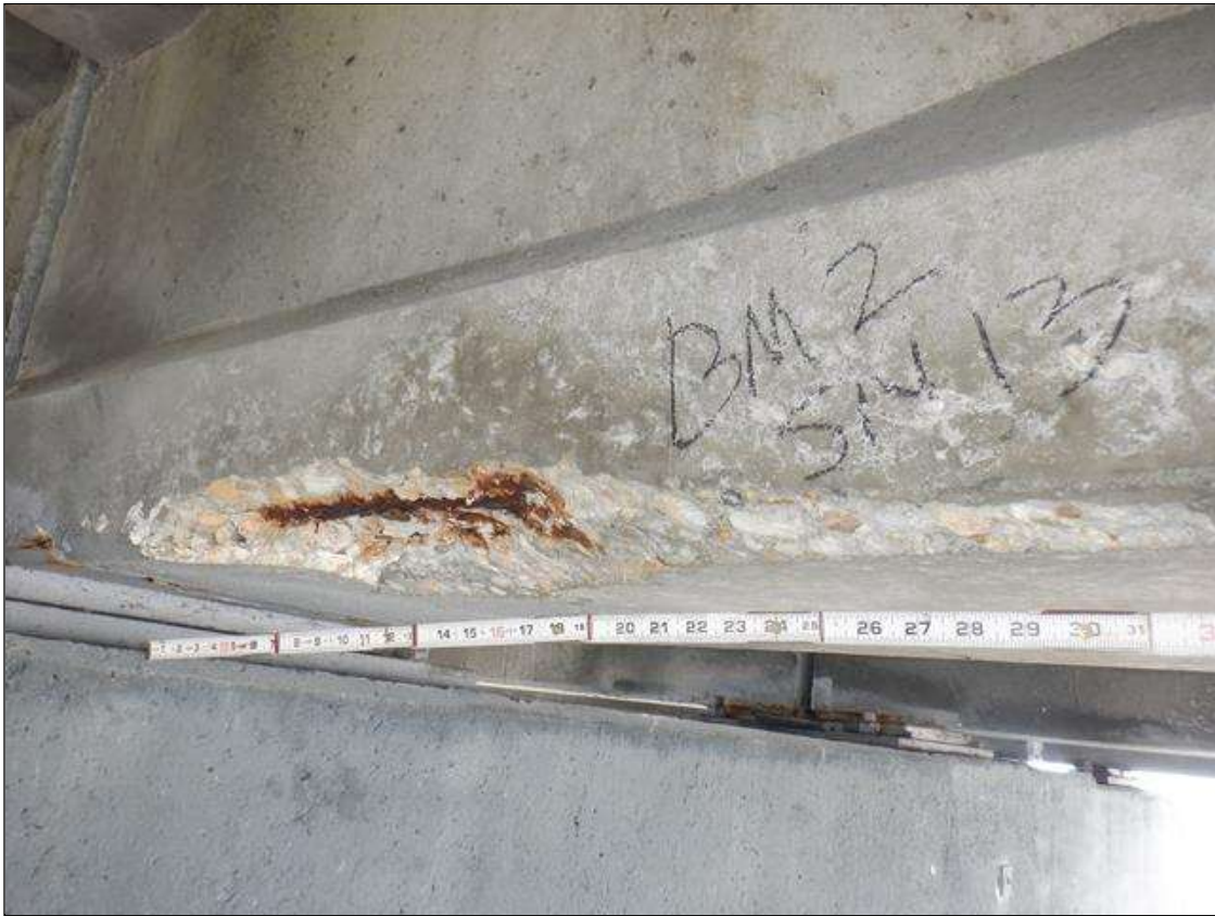
Span 13 Beam 2: (PAR) BOTTOM FLANGE NORTH FACE, AT BENT 13, SPALL (34 INCHES X 8 INCHES X 2 INCHES DEEP) WITH EXPOSED RUSTED STRANDS (20 PERCENT SECTION LOSS)
