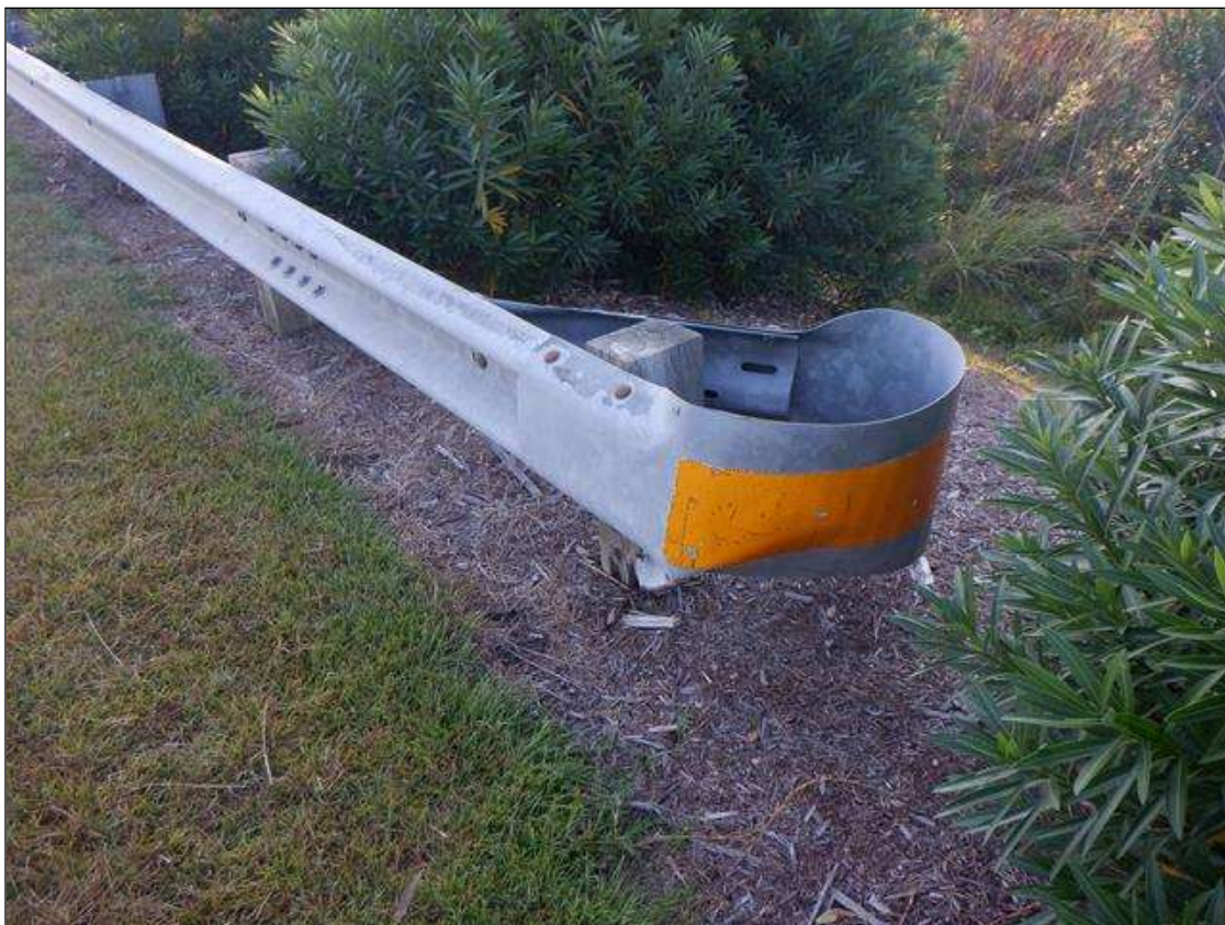
SOUTHWEST GUARDRAIL END TREATMENT
