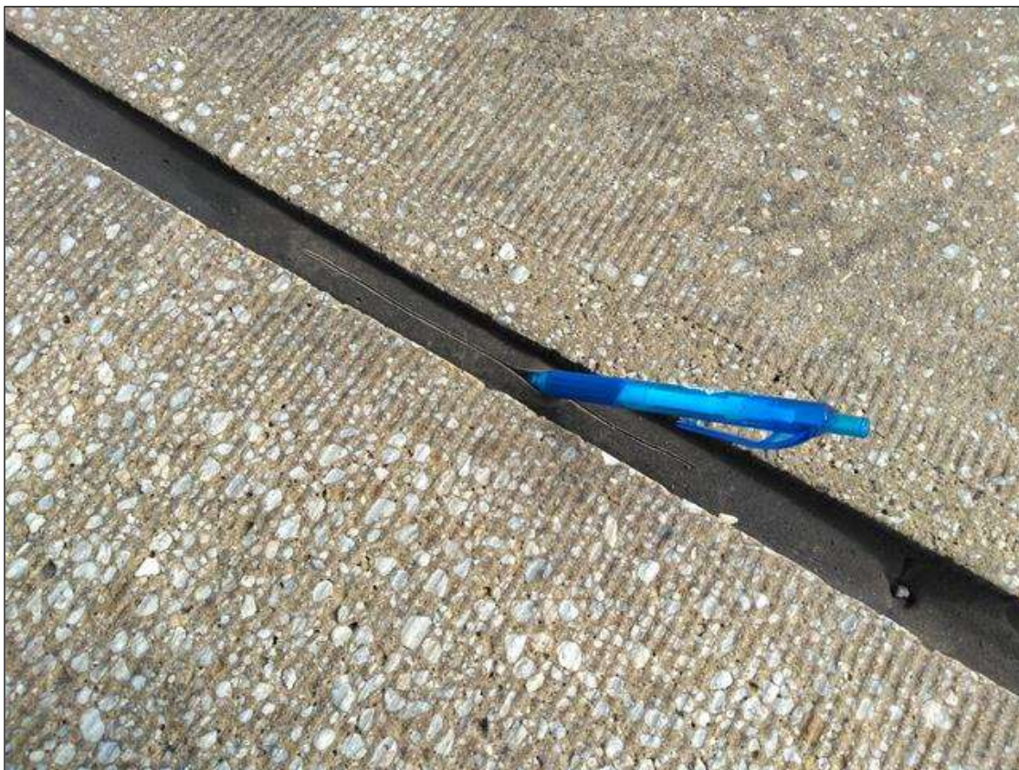
Span 28 Expansion Joint Bent 27: LEFT LANE, PARTIAL DEPTH SEAL DAMAGE (14 FEET)
