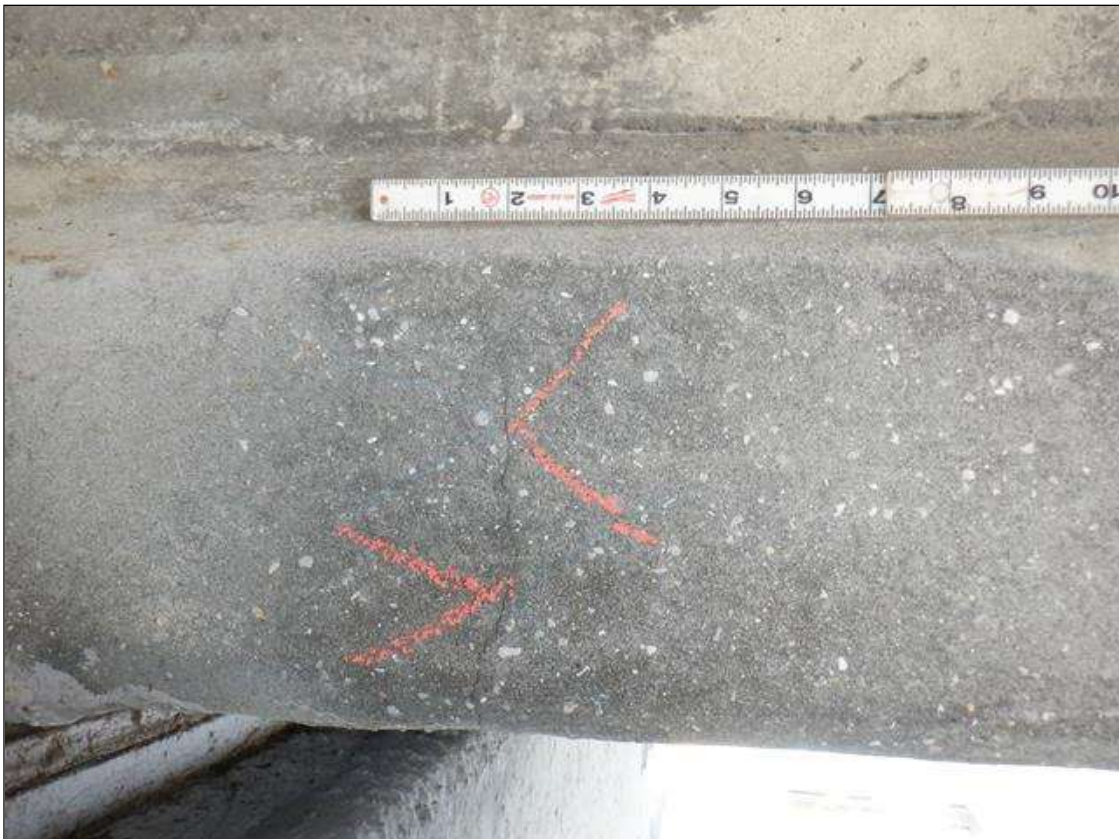
Span 6 Beam 2: SOUTH FACE OF BOTTOM FLANGE AT BENT 5, VERTICAL CRACK (6INCHES LONG X UP TO 0.015 INCHES)
