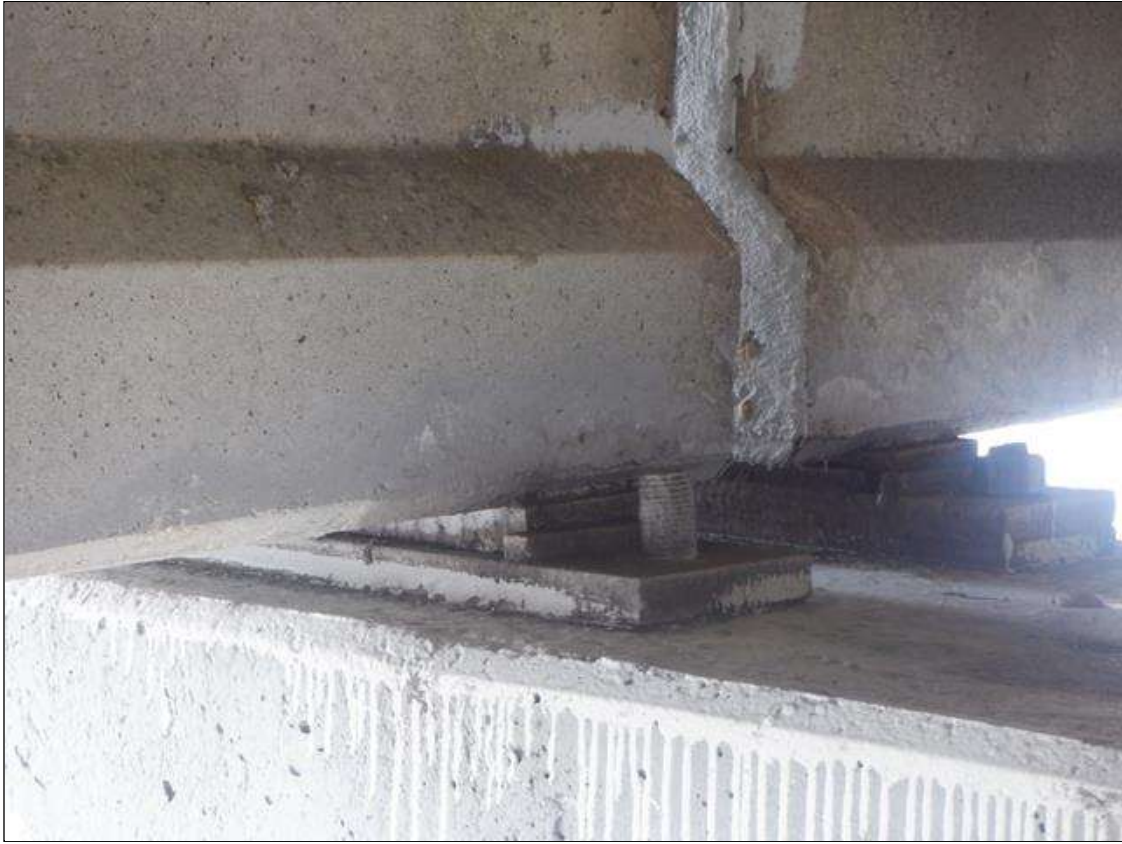
Span 191 Near Bearing: (PAR) AT NORTH FACE, MISSING ANCHOR BOLT NUT
