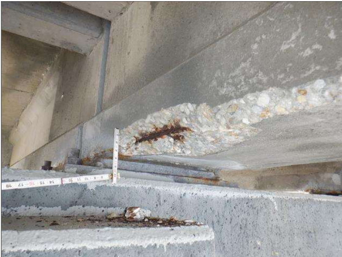
Span 52 Beam 2: (PAR) NORTH FACE OF BOTTOM FLANGE AT 1FEET FROM BENT 52, SPALL (29INCHES X UP TO 6INCHES X 2IN) WITH EXPOSED STRAND (10 PERCENT SECTION LOSS)
