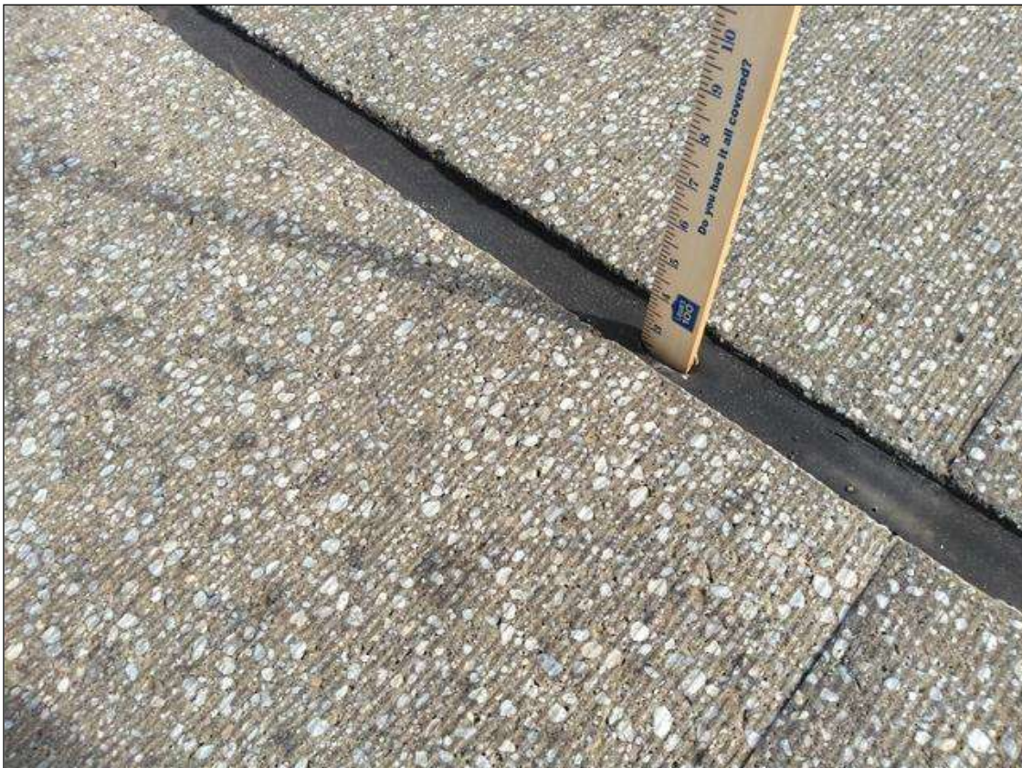
Span 26 Expansion Joint Bent 25: AT BENT 25, SEAL CRACKING UP TO 6 INCH TOTAL ACROSS 3 LOCATIONS IN RIGHT LANE
