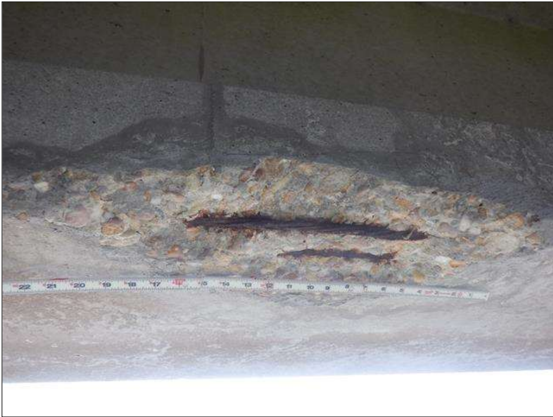
Span 171 Beam 4: (PAR) NORTH FACE OF BOTTOM FLANGE AT 10 FEET FROM BENT 171, SPALL (20 INCHES X 8 INCHES X 2 INCHES) WITH TWO (2) EXPOSED STRANDS (50 PERCENT SECTION LOSS) ON STRAND
