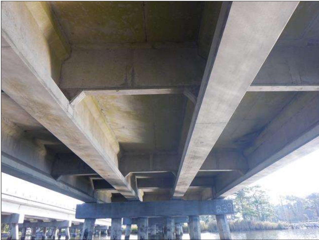
TYPICAL SUPERSTRUCTURE FRAMING, TYPICAL UNDERSIDE OF DECK (SPAN 239 IN VIEW)
