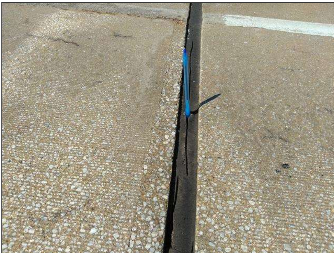
Span 196 Expansion Joint Bent 195: AT BENT 195, PARTIAL DEPTH CRACKING INTERMITTENT THROUGHOUT
