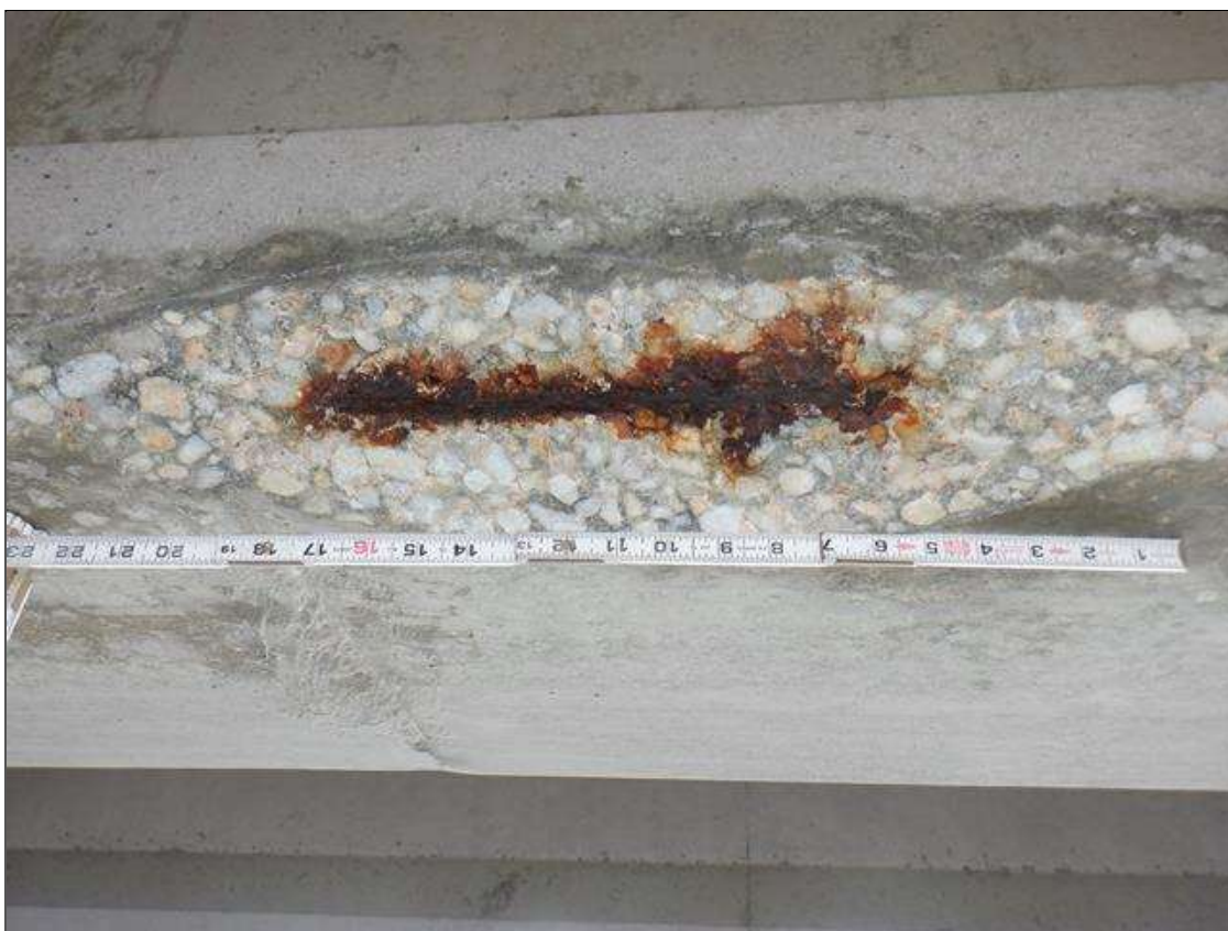
Span 203 Beam 2: (PAR) NORTH FACE AND UNDERSIDE OF BOTTOM FLANGE AT MIDSPAN, SPALL (26 INCHES LONG X 5 INCHES WIDE X 2 INCHES DEEP) WITH EXPOSED RUSTED STRANDS (20 PERCENT SECTION LOSS)
