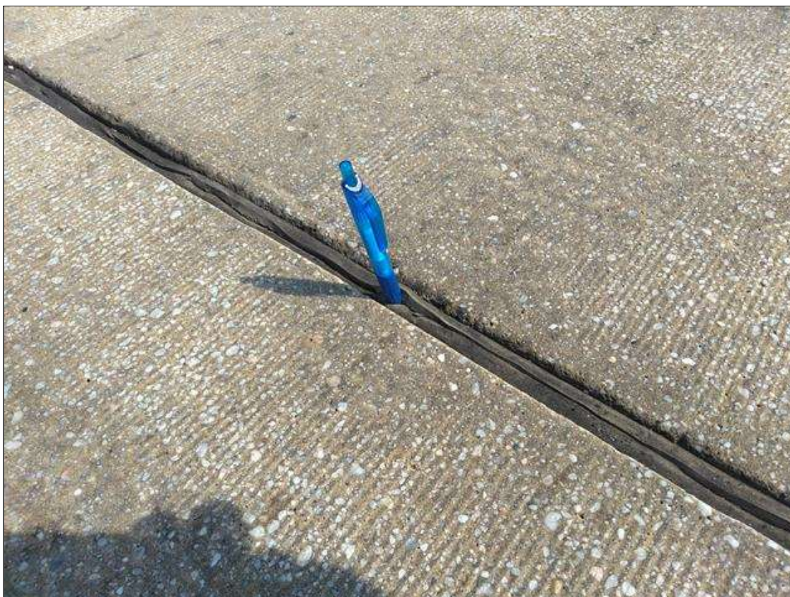
Span 151 Expansion Joint Bent 150: FULL WIDTH, SEAL DAMAGED AND TORN (24 FEET)
