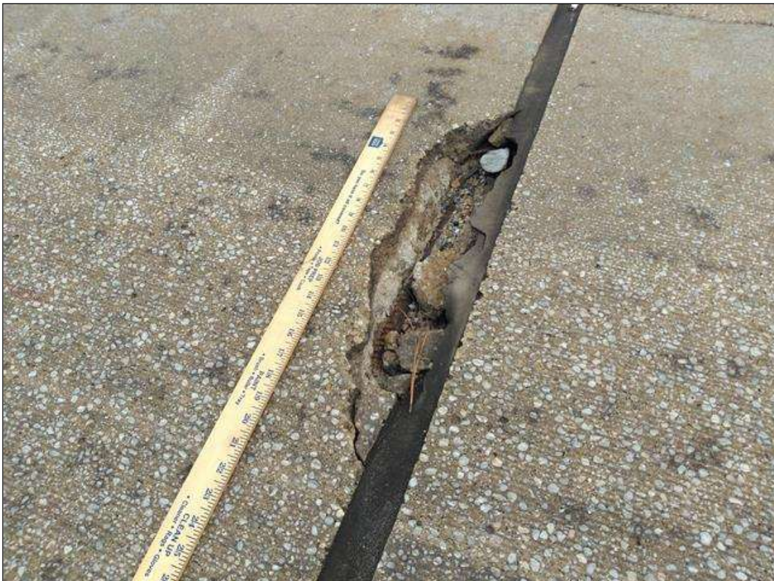
Span 77 Expansion Joint Bent 76: (PAR) AT BENT 76, RIGHT LANE SPALL WITH EXPOSED REINFORCEMENT WITH CORROSION. 2 FEET WIDE X 4 INCHES LONG X 3 INCHES DEEP.
