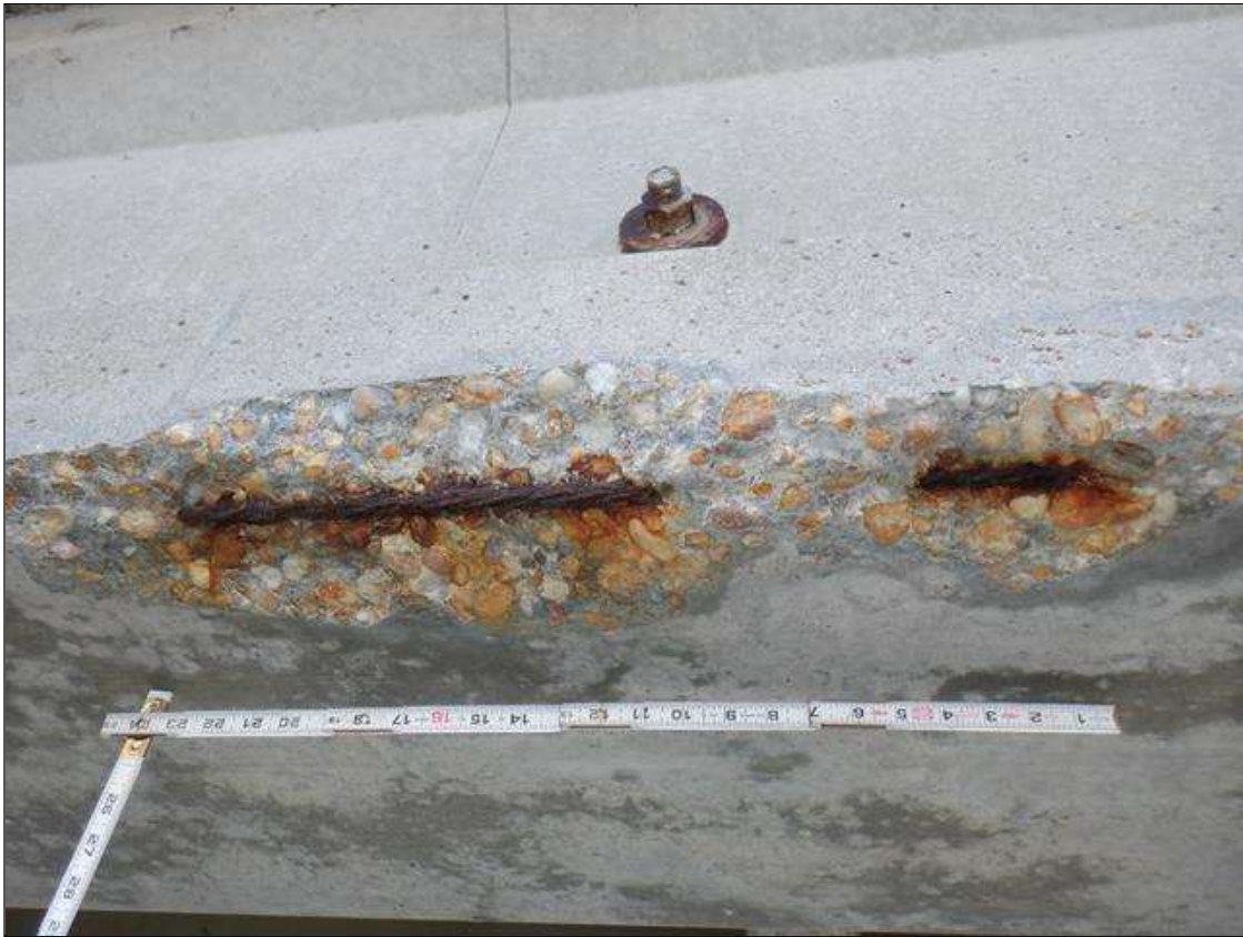
Span 162 Beam 1: (PAR) NORTH FACE OF BOTTOM FLANGE AT 20 FEET FROM BENT 161, SPALL (30 INCHES X 6 INCHES X 3 INCHES) WITH EXPOSED STRANDS (5 PERCENT SECTION LOSS) ON STRAND
