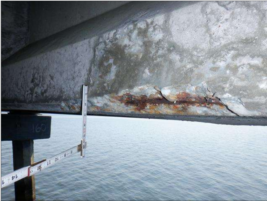
Span 160 Beam 3: (PAR) NORTH FACE OF BOTTOM FLANGE, AT 22FEET FROM BENT 160, SPALL (24INCHES X 6INCHES X 2 INCHES) WITH EXPOSED STRANDS (5 PERCENT SECTION LOSS) ON STRAND
