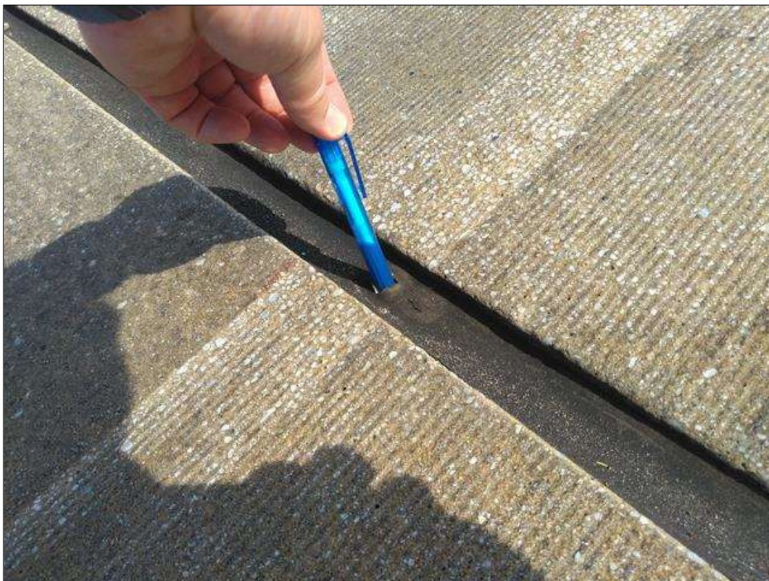
Span 134 Expansion Joint Bent 133: AT BENT 133, 2 INCH WIDE X FULL DEPTH CRACK IN RIGHT LANE
