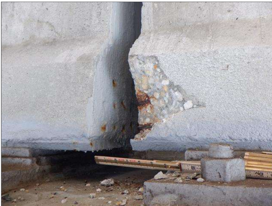
Span 219 Beam 3: SOUTH FACE OF BOTTOM FLANGE AT BENT 218, SPALL (6 INCHES LONG X 7 INCHES HIGH X 2 INCHES DEEP) WITH EXPOSED RUSTED REINFORCING (NO MEASURABLE SECTION LOSS)
