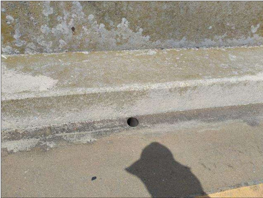
Span 65 Left Bridge Rail: CURB AT 6FEET FROM BENT 64, SPALL (4INCHES X 6INCHES X 1/2 INCHES) WITH EXPOSED RUSTED REBAR (DEFECT NOT FOUND 9/12/22)
