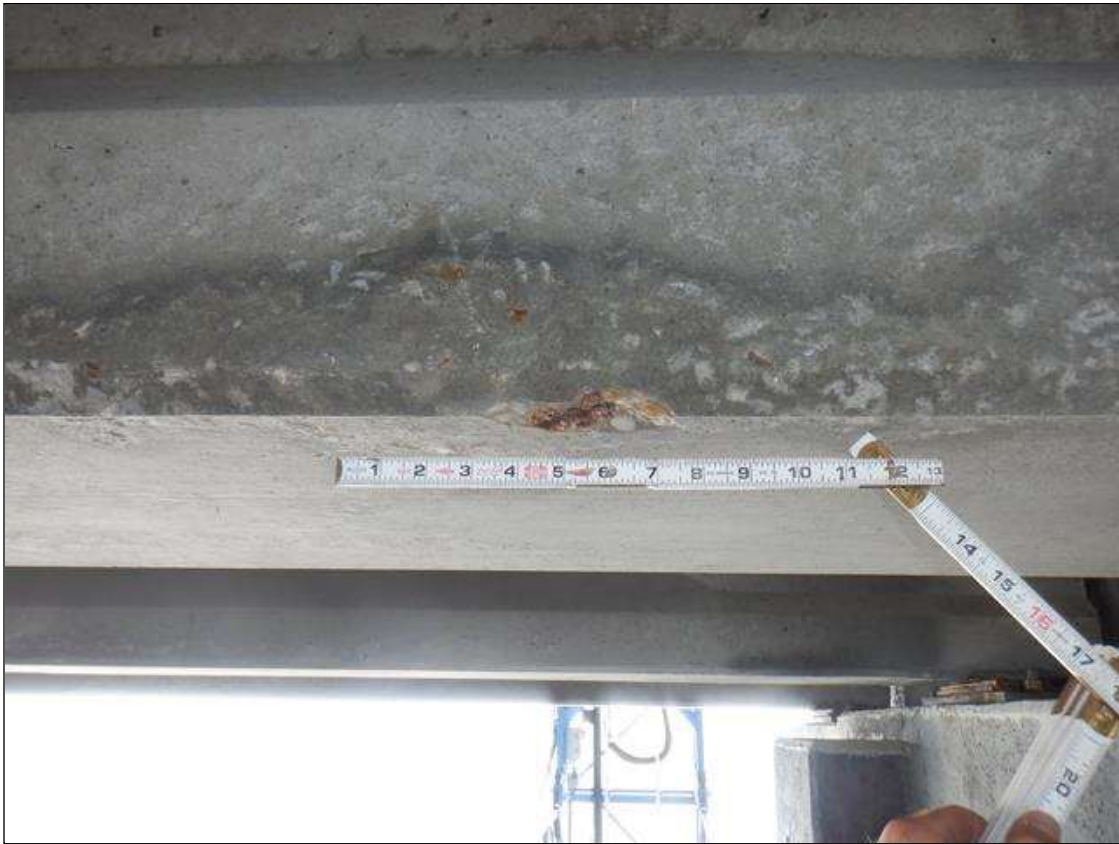
Span 29 Beam 2: BOTTOM FLANGE NORTH FACE, 3 FEET FROM BENT 28 HORIZONTAL CRACK (HAIRLINE X 6 INCHES LONG) WITH RUST STAIN AND SPALL/DELAMINATION (2 INCHES X 1 INCH X 1/2 INCH DEEP) WITH EXPOSED RUSTED REINFORCING (NO LOSS)
