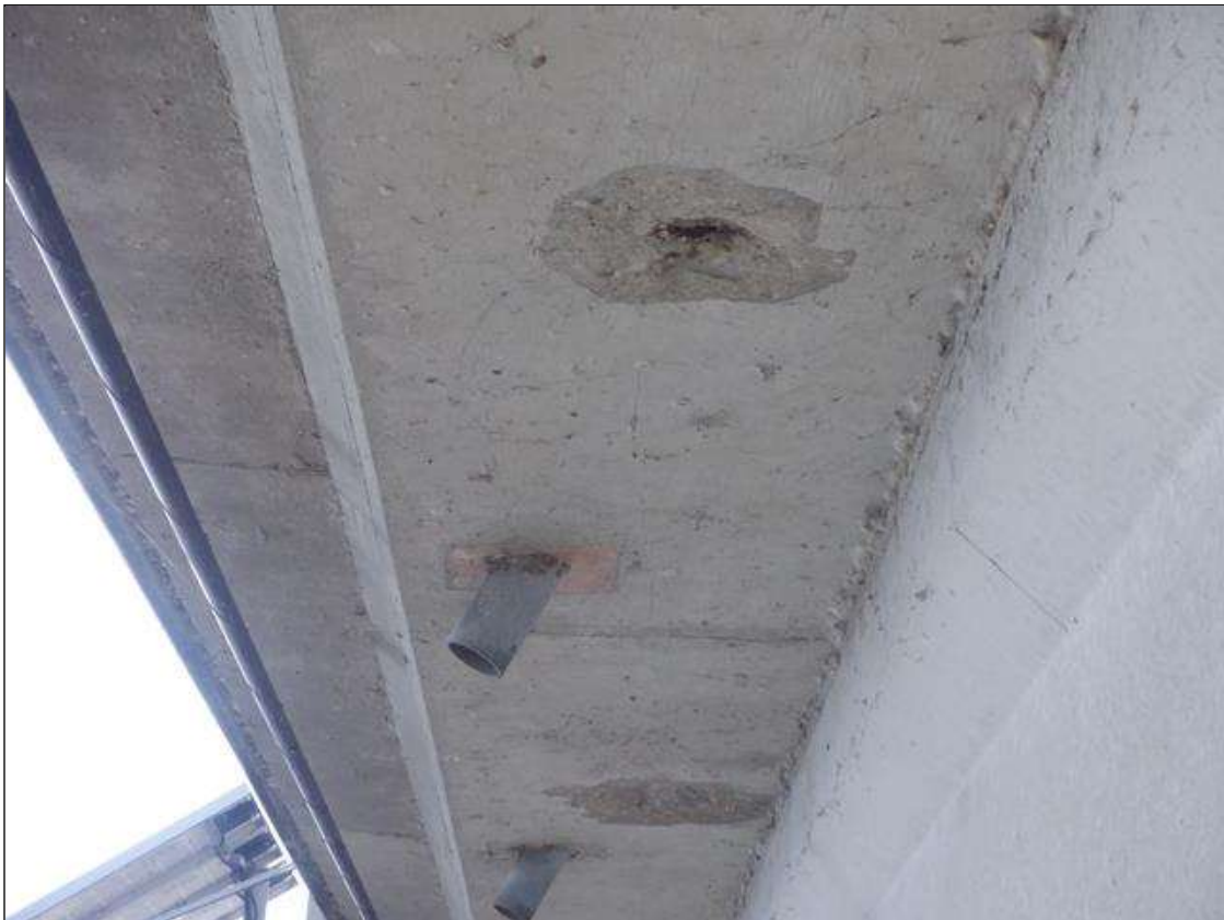
Span 180 Deck: UNDERSIDE OF DECK SOUTH OVERHANG AT MIDSPAN, (2) SPALLS (UP TO 16 INCHES DIAMETER X 2 INCHES) WITH EXPOSED RUSTED REBAR
