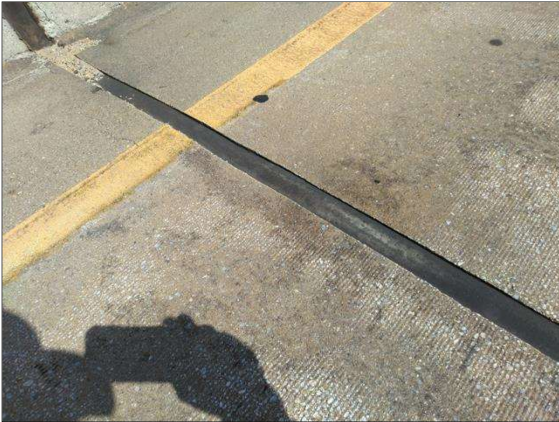
Span 44 Expansion Joint Bent 43: 1 FEET LONG AREA OF FULL DEPTH LOSS OF ADHESION STARTING 3 FEET FROM LEFT RAIL INCHES LEFT EASTBOUND TRAVEL LANE OVER PIER 43. (DEFECT NOT FOUND 9/12/22)
