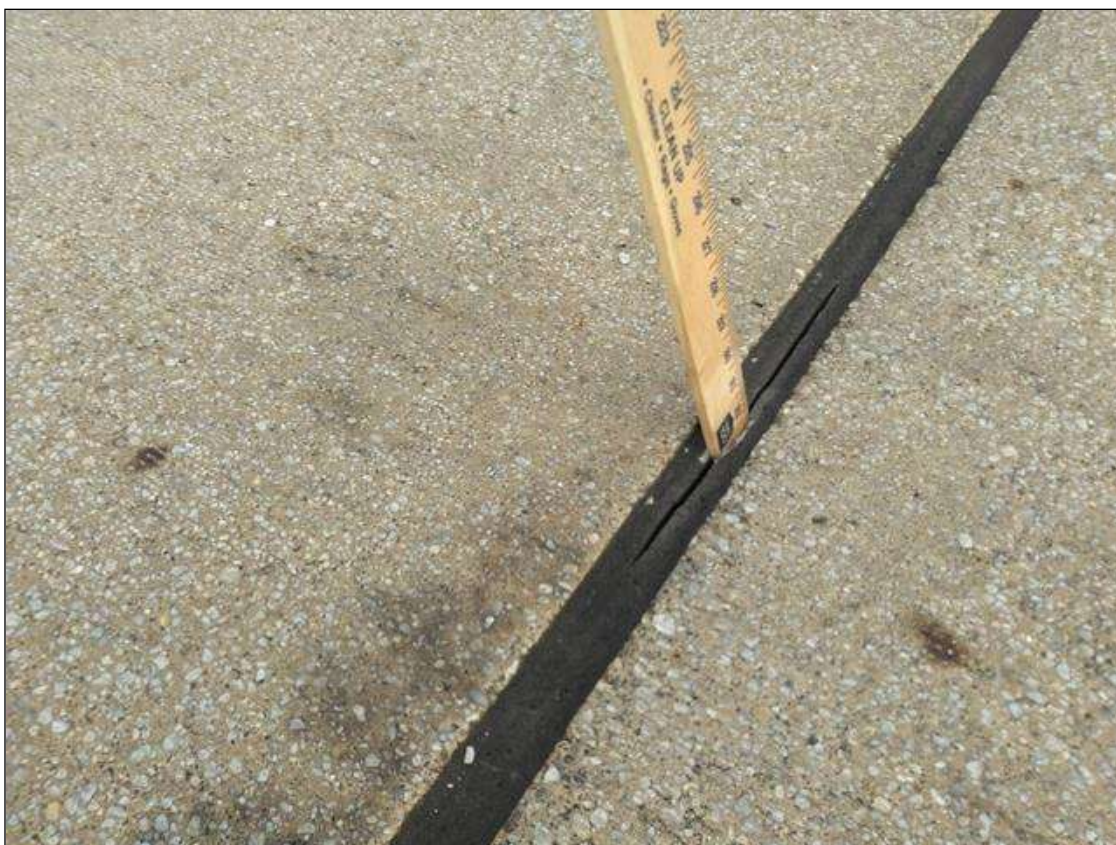
Span 103 Expansion Joint Bent 102: MIDDLE OF LEFT LANE, SEAL DAMAGE (2 FEET)
