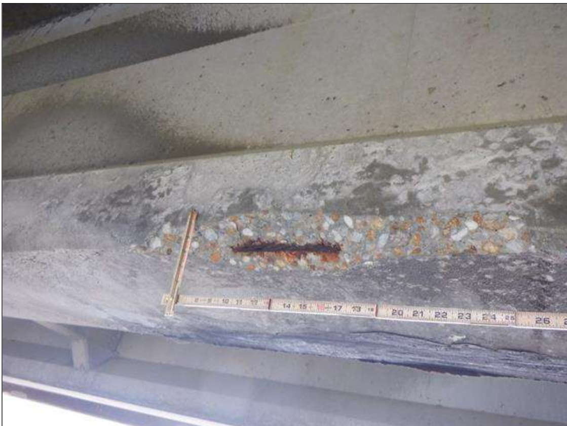
Span 114 Beam 2: (PAR) NORTH FACE OF BOTTOM FLANGE AT MIDSPAN, SPALL (26 INCHES LONG X 3 INCHES HIGH X 2 INCHES DEEP) WITH (1) EXPOSED STRAND (5 PERCENT LOSS)
