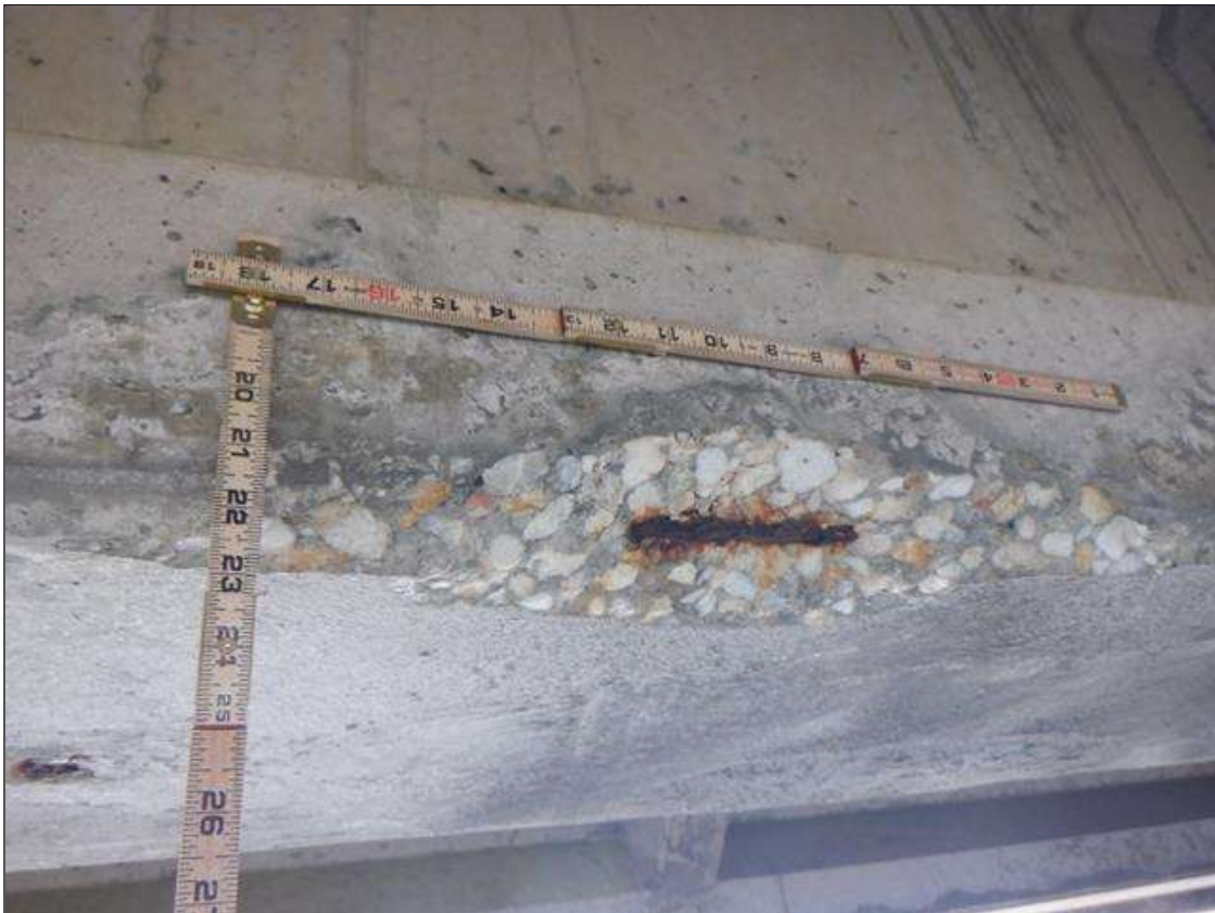
Span 229 Beam 2: (PAR) NORTH FACE OF BOTTOM FLANGE AT 22 FEET FROM BENT 228, SPALL (18 INCHES X 5 INCHES X 2 INCHES) WITH EXPOSED STRAND (10 PERCENT SECTION LOSS) ON STRAND
