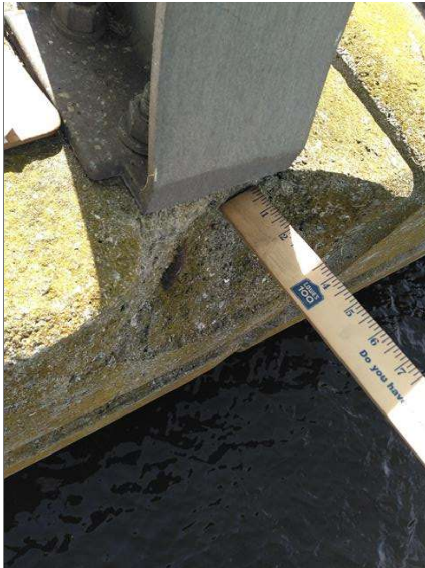
Span 57 Left Bridge Rail: BACK OF RAIL AT POST 1, 12 INCH LONG X 9 INCH HIGH X 2.5 INCH DEEP SPALL WITH EXPOSED REBAR WITH CORROSION
