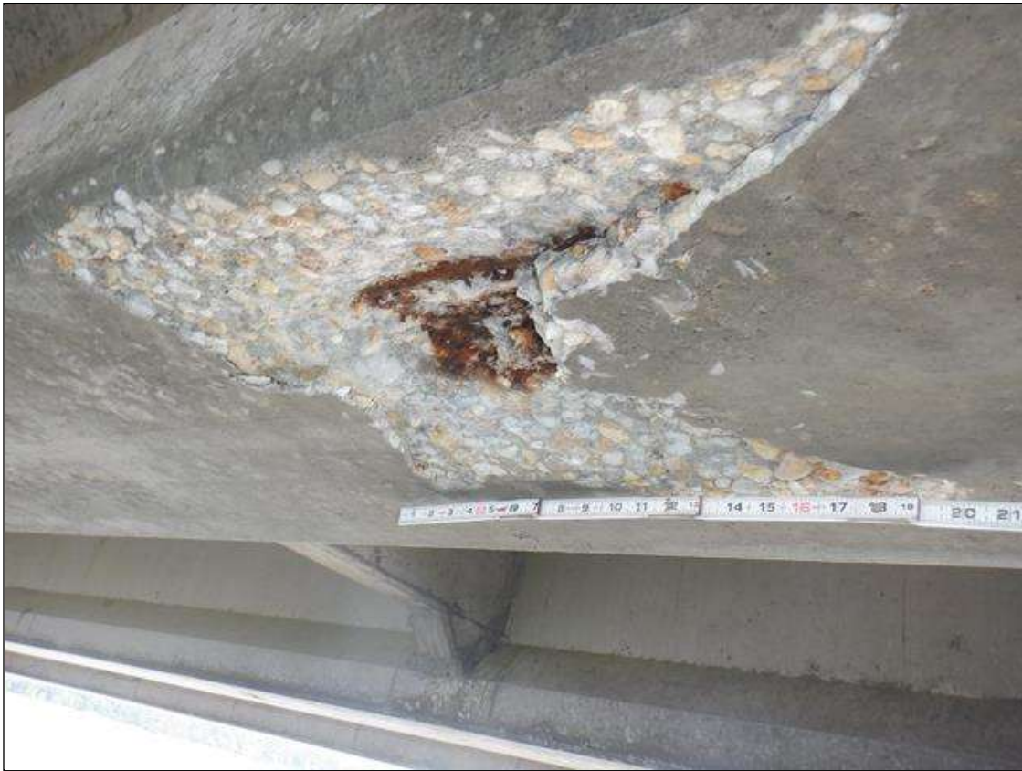
Span 210 Beam 2: (PAR) BOTTOM OF BOTTOM FLANGE AT 10 FEET FROM BENT 209, SPALL (18 INCHES LONG X 5 INCHES WIDE X 1.5 INCHES DEEP) WITH EXPOSED RUSTED STRANDS (10 PERCENT SECTION LOSS)
