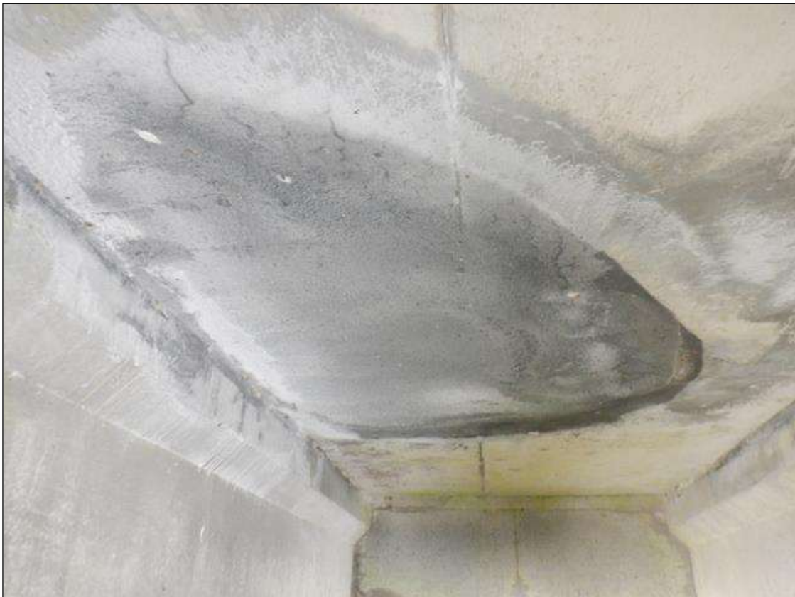
Span 1 Deck: UNDERSIDE OF DECK, BAY 2 NEXT TO GIRDER 3, PATCHED AREA (8 FEET X 5 FEET)
