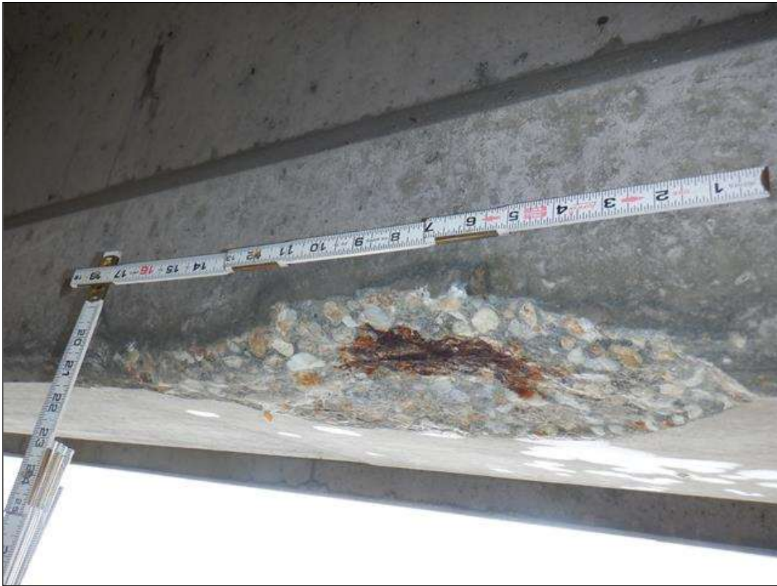
Span 59 Beam 3: (PAR) BOTTOM FLANGE NORTH FACE AT 12 FEET FROM BENT 58, SPALL (18 INCHES LONG X 7 INCHES WIDE X UP TO 2 INCHES DEEP) WITH EXPOSED RUSTED STRANDS (30 PERCENT SECTION LOSS)
