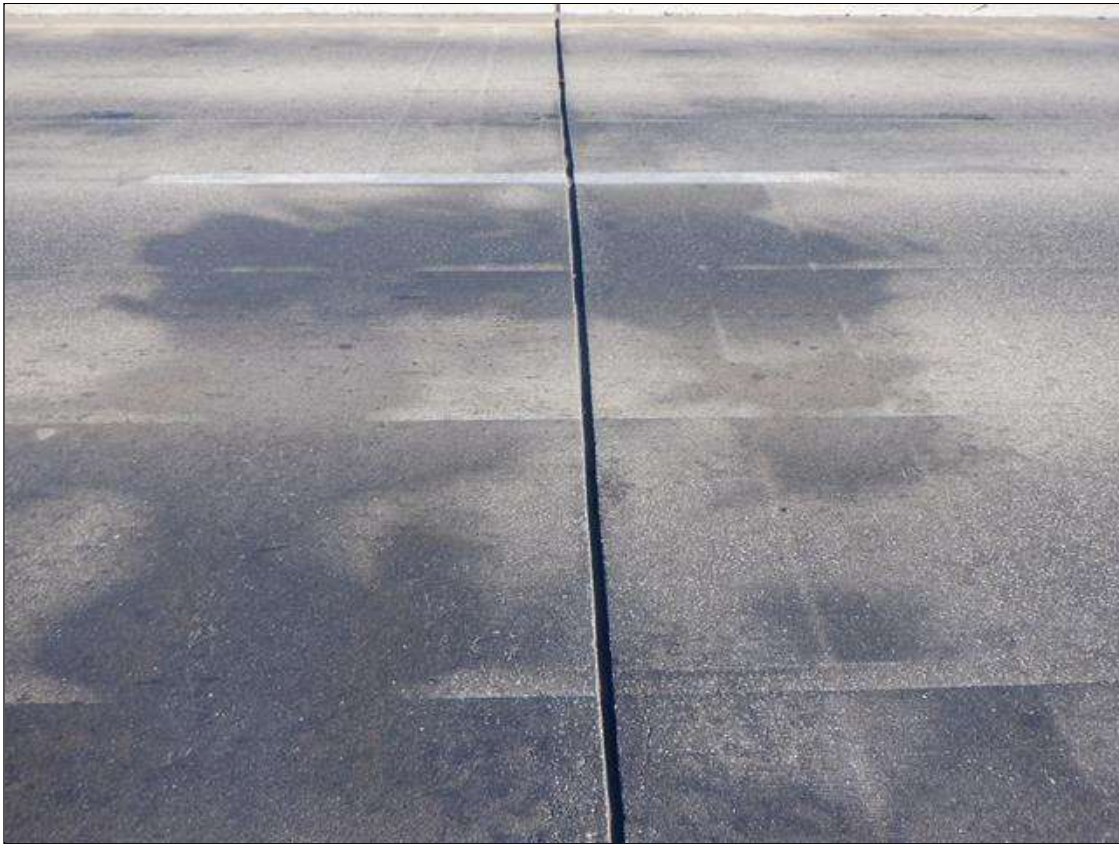
TYPICAL JOINT OVER INTERIOR BENT, JOINT OVER BENT 1 IN VIEW
