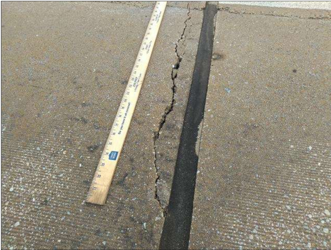
Span 70 Expansion Joint Bent 69: EXTENDING 4 FEET FROM RIGHT SHOULDER AT BENT 69, CRACK UP TO 0.50 INCH WIDE RUNNING 3 INCHES FROM JOINT UP TO 1.5 INCH DEEP
