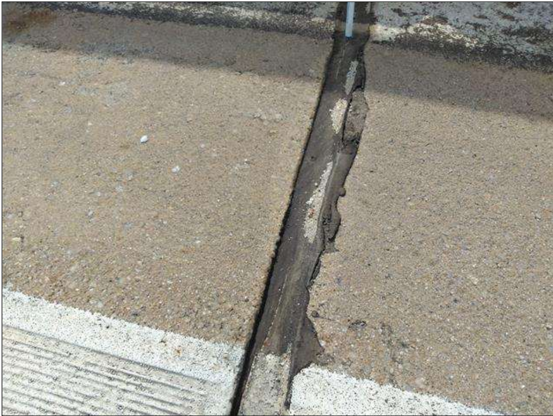
Span 241 Expansion Joint Bent 240: AT BENT 240, PARTIAL DEPTCH CRACKS IN BOTH SHOULDERS AND AT CENTER
