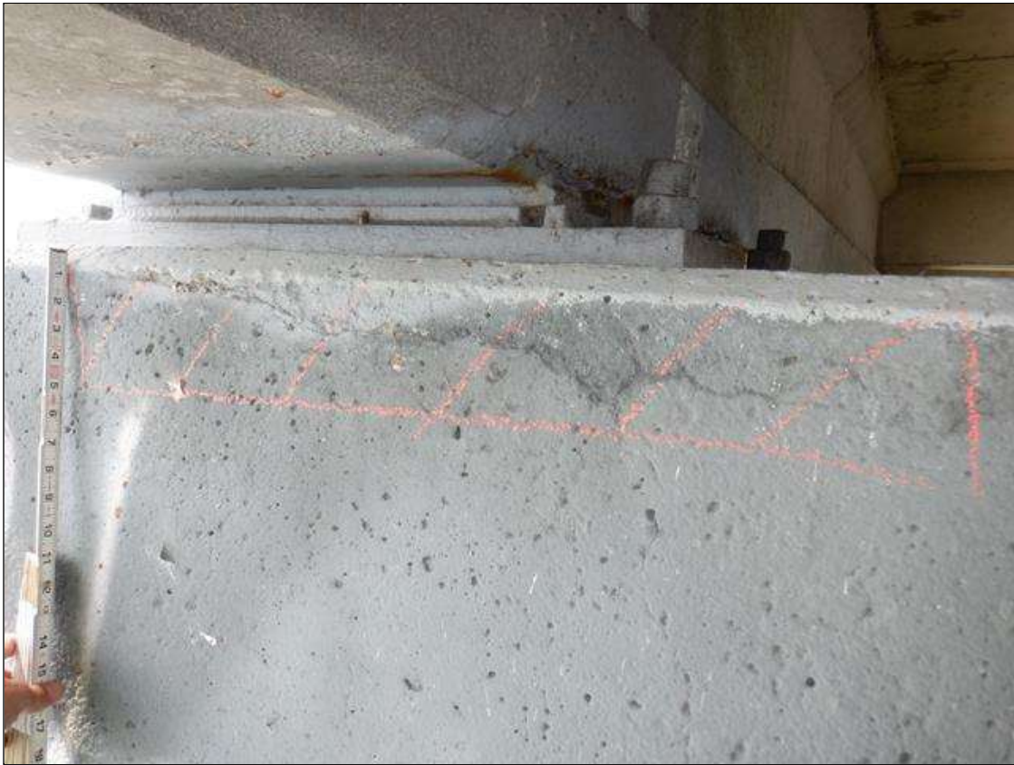
Bent 36 Cap 1: TOP OF EAST FACE AT BEAM 4, DELAMINATION (28 INCHES LONG X 5 INCHES HIGH)
