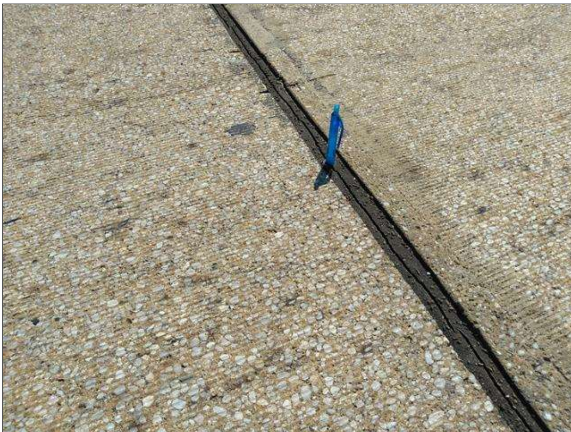
Span 182 Expansion Joint Bent 181: AT BENT 181, FULL WIDTH AND DEPTH CRACKING
