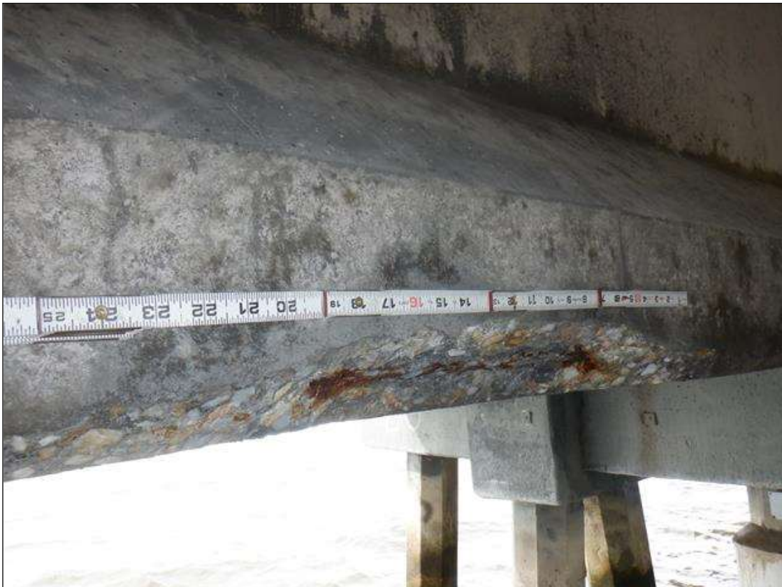
Span 81 Beam 2: (PAR) BOTTOM FLANGE NORTH FACE AT 16 FEET FROM BENT 80, FAILED PATCH/SPALL (24 INCHES X 4 INCHES X 2 INCHES DEEP) WITH EXPOSED RUSTED STRANDS (30 PERCENT SECTION LOSS)
