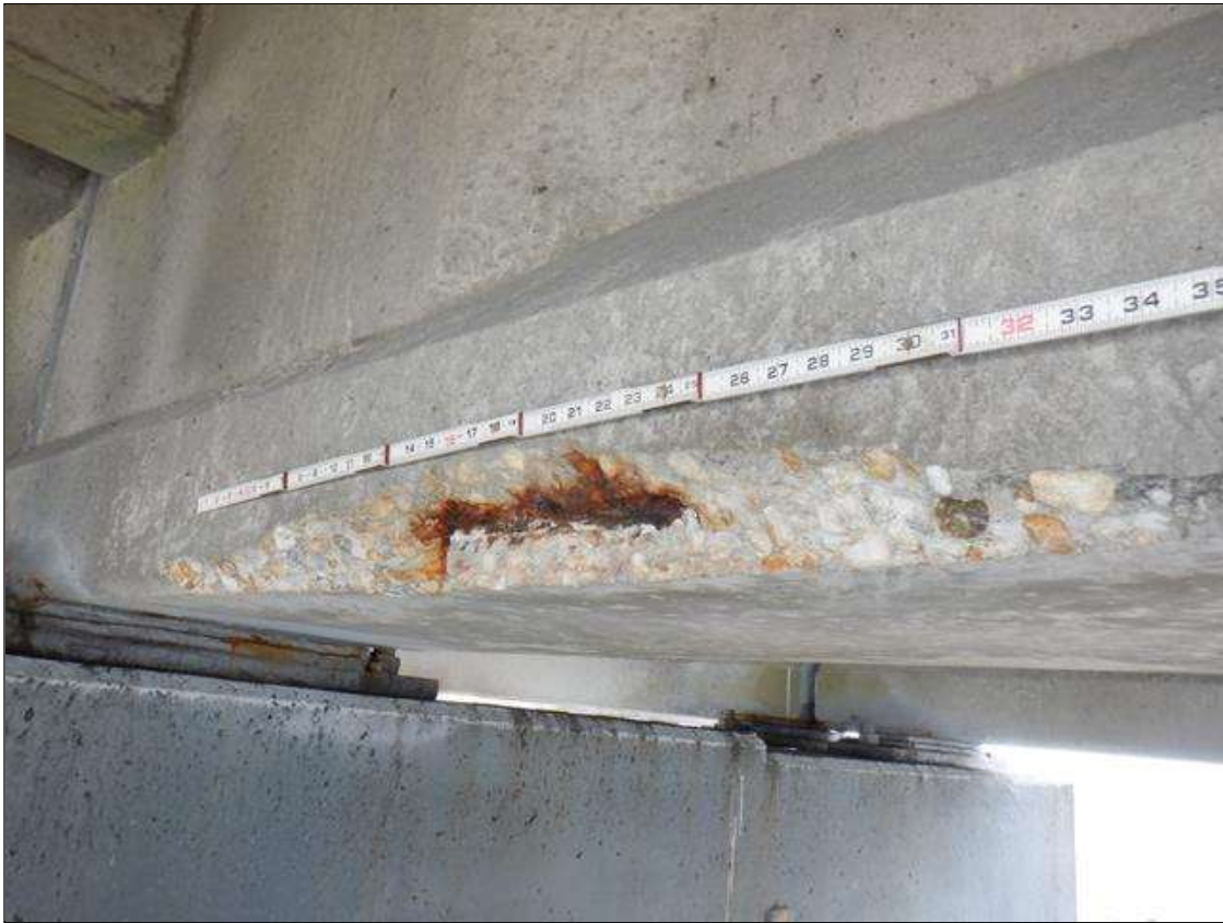
Span 67 Beam 2: (PAR) BOTTOM FLANGE SOUTH FACE AT 2 FEET FROM BENT 67, SPALL (36 INCHES LONG X 4 INCHES HIGH X 2 INCHES DEEP) WITH EXPOSED RUSTED STRANDS (10 PERCENT SECTION LOSS)
