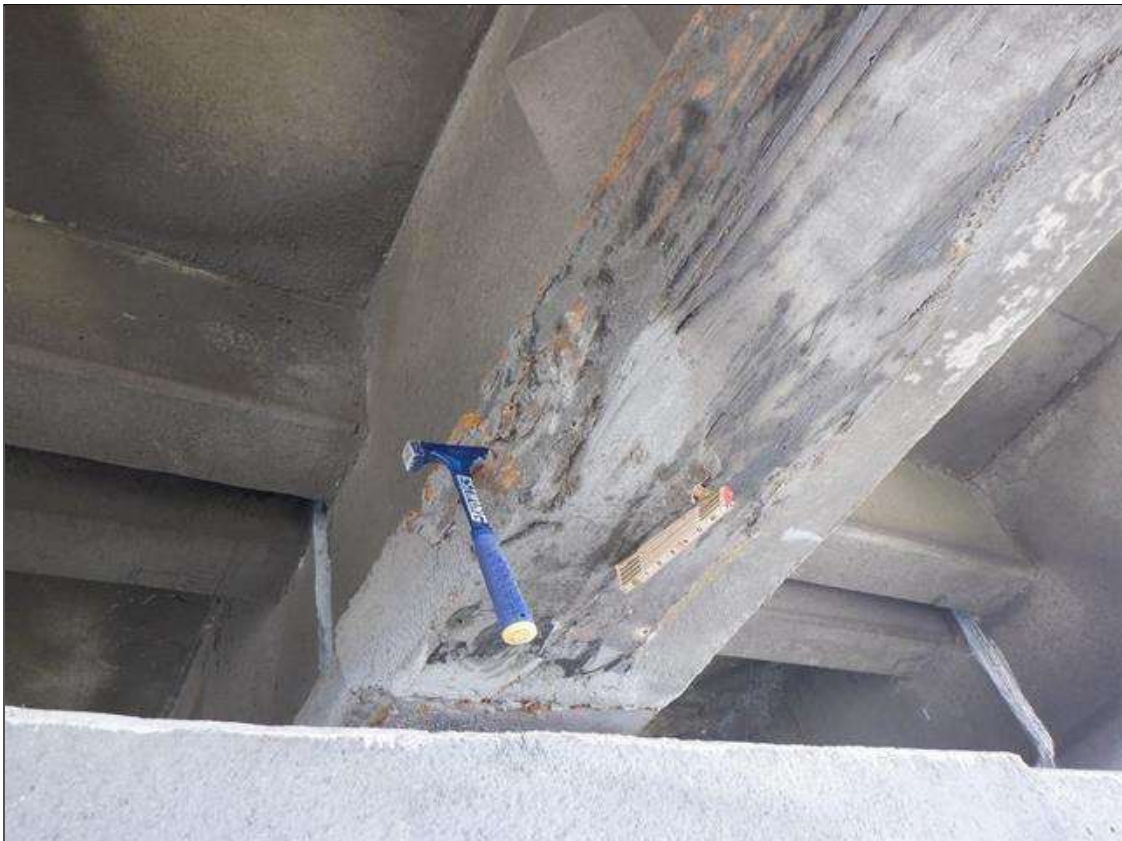
Span 134 Beam 3: (PAR) NORTH FACE AND BOTTOM OF BOTTOM FLANGE AT BENT 134, DELAMINATION (32 INCHES LONG X 7 INCHES HIGH X 10 INCHES WIDE) WITH CRACKS (UP TO 1/2 INCH WIDE)
