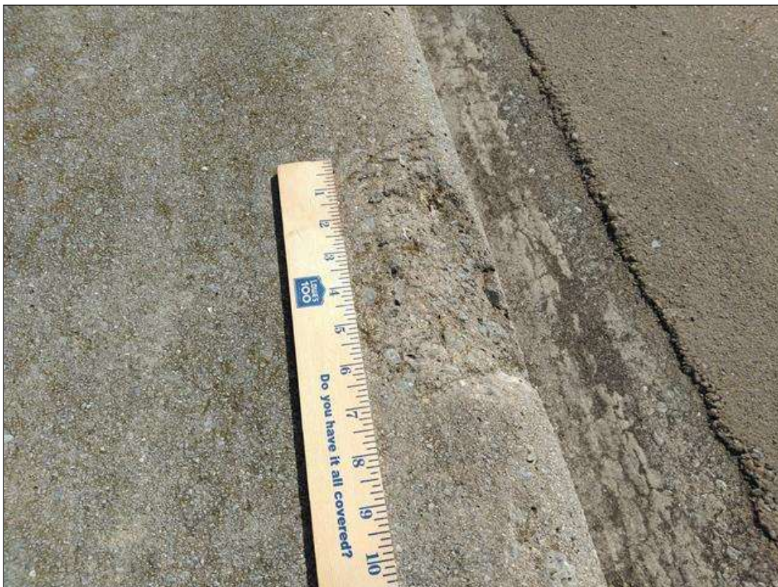
Span 21 Left Bridge Rail: CURB AT RAILPOST 3, SPALL (8INCHES X 4INCHES X 1 INCHES)
