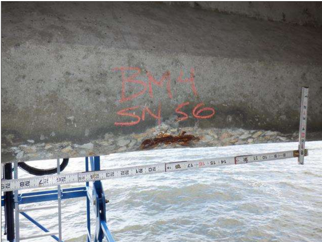
Span 56 Beam 2: (PAR) BOTTOM FLANGE NORTH FACE NEAR MIDSPAN, SPALL (24 INCHES LONG X 2 INCHES HIGH X 2 INCHES DEEP) WITH EXPOSED RUSTED STRANDS (5 PERCENT SECTION LOSS)
