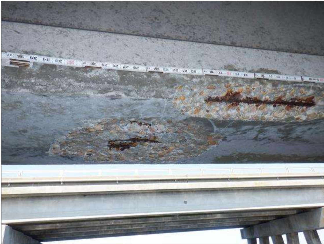
Span 163 Beam 1: (PAR) SOUTH FACE OF BOTTOM FLANGE AT 18 FEET FROM BENT 162, (2) TWO SPALLS (40 INCHES X FULL WIDTH X 2 INCHES DEEP) WITH (5) FIVE EXPOSED RUSTED STRANDS (10 PERCENT SECTION LOSS) ON STRAND
