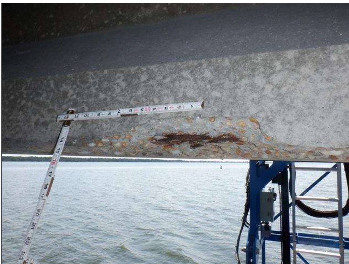
Span 162 Beam 4: (PAR) NORTH FACE OF BOTTOM FLANGE AT 12 FEET FROM BENT 161, SPALL (24 INCHES X 8 INCHES X 3 INCHES) WITH EXPOSED STRANDS (20 PERCENT SECTION LOSS) ON STRAND
