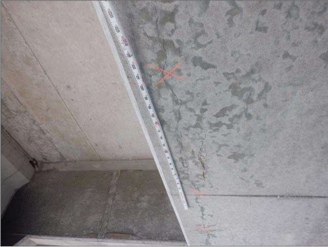
Span 174 Beam 3: BOTTOM OF BOTTOM FLANGE 20 FEET FROM BENT 174, LONGITUDINAL CRACK (10 FEET LONG X UP TO 0.012 INCHES WIDE) WITH ASSOCIATED EDGE SPALLING
