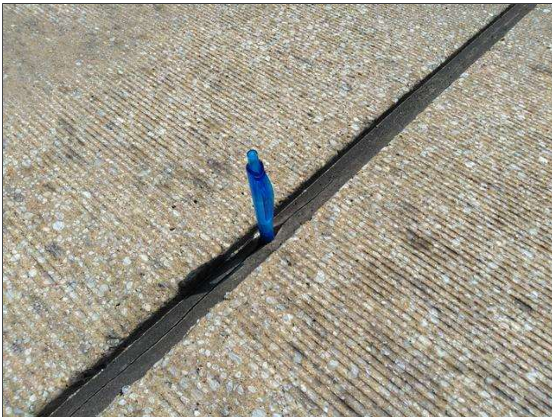
Span 166 Expansion Joint Bent 165: AT BENT 165, INTERMITTENT FULL DEPTH CRACKING THROUGHOUT
