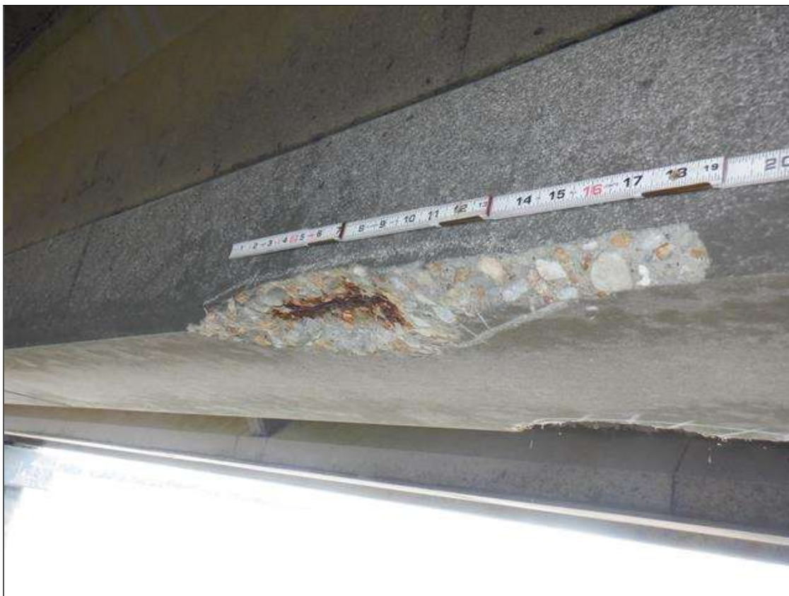
Span 163 Beam 2: (PAR) BOTTOM FLANGE, NORTH AND BOTTOM FACES, 7 FEET FROM BENT 162, SPALL (21 INCHES LONG X 5 INCHES HIGH X 1 INCH DEEP) WITH EXPOSED RUSTED STRANDS (10 PERCENT SECTION LOSS)
