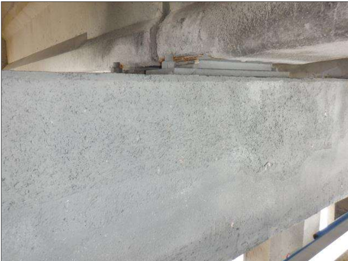
Bent 15 Cap 1: 4 FEET LONG X 1.25 FEET HIGH DELAMINATION ON TOP OF CAP UNDER BEAM 3
