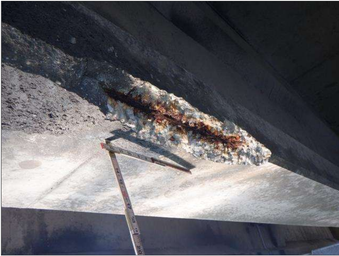
Span 221 Beam 3: (PAR) NORTH FACE OF BOTTOM FLANGE AT 20 FEET BENT 220, FAILED PATCHED/SPALL (30 INCHES X 2.5 INCHES HIGH X 4 INCHES WIDE X 1.5 INCH DEEP) WITH EXPOSED RUSTED STRANDS (20 PERCENT SECTION LOSS)
