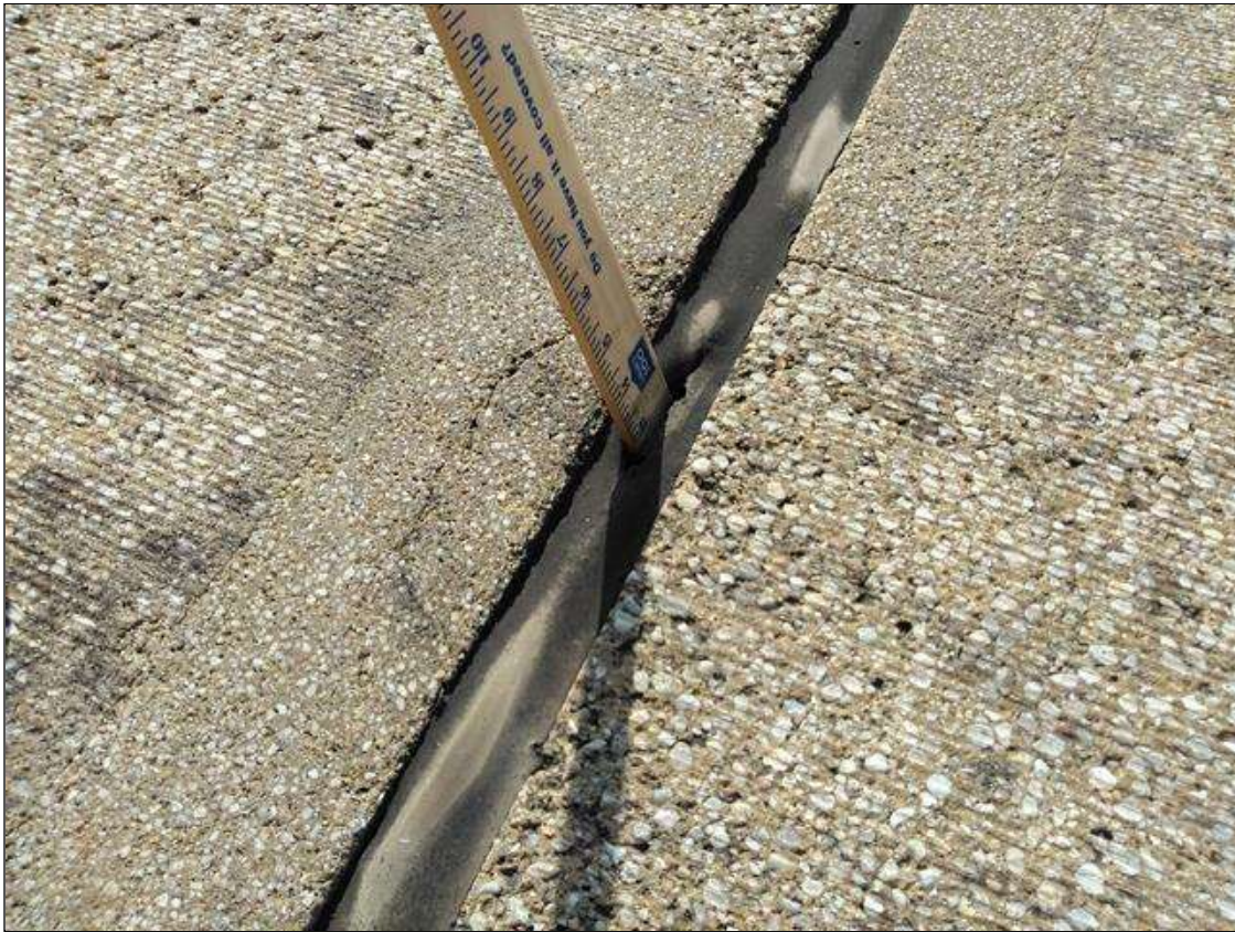
Span 25 Expansion Joint Bent 24: BENT 24 JOINT, CRACK IN LEFT LANE, 3 INCH LONG X FULL DEPTH
