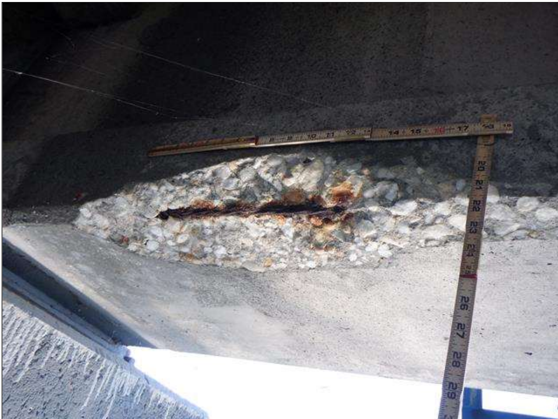
Span 233 Beam 4: (PAR) NORTH FACE OF BOTTOM FLANGE, AT 2 FEET FROM BENT 233, SPALL (30 INCHES X 6 INCHES X 2 INCHES) WITH EXPOSED STRAND (10 PERCENT SECTION LOSS) ON STRAND
