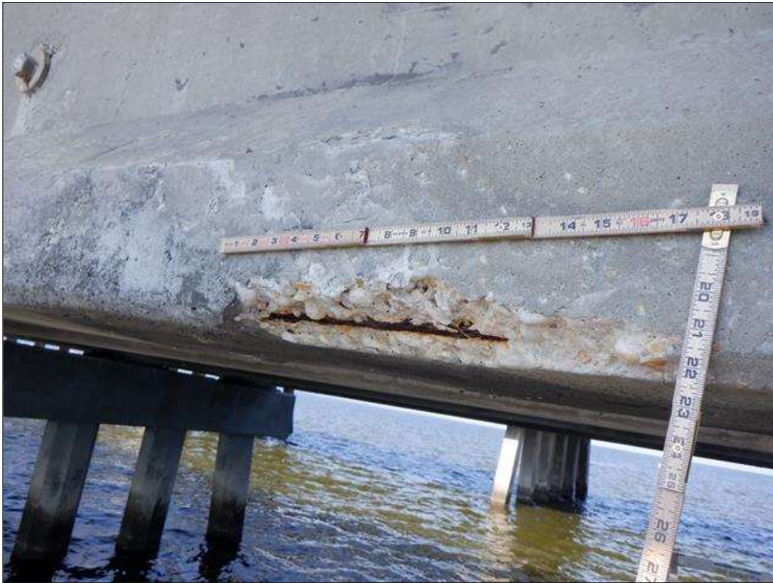
Span 229 Beam 4: (PAR) SOUTH FACE OF BOTTOM FLANGE AT 22 FEET FROM BENT 228, SPALL (18 INCHES X 5 INCHES X 2 INCHES) WITH EXPOSED STRAND (10 PERCENT SECTION LOSS)
