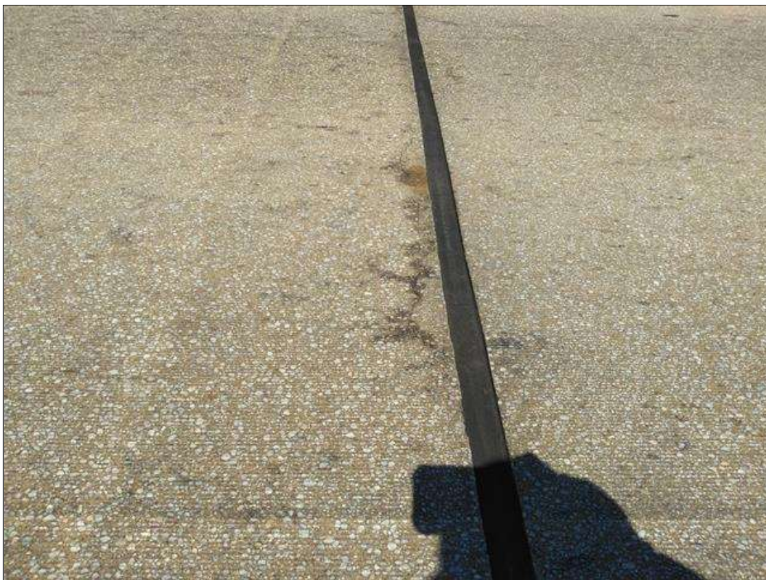
Span 55 Expansion Joint Bent 54: MIDDLE OF LANE, DELAMINATION (3FEET X 3 INCHES)
