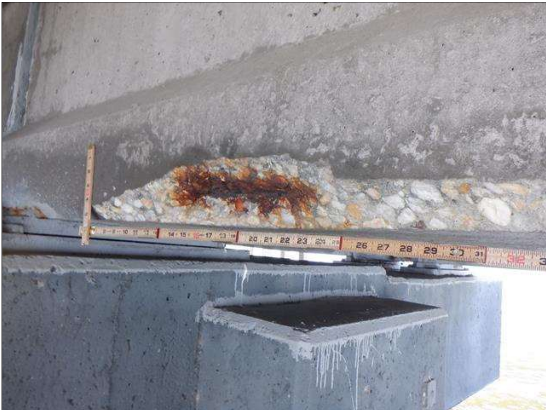
Span 223 Beam 2: (PAR) BOTTOM FLANGE SOUTH FACE AT 2 FEET FROM BENT 222, SPALL (38 INCHES LONG X 4 INCHES HIGH X 2 INCHES DEEP) WITH EXPOSED RUSTED STRANDS (20 PERCENT SECTION LOSS)
