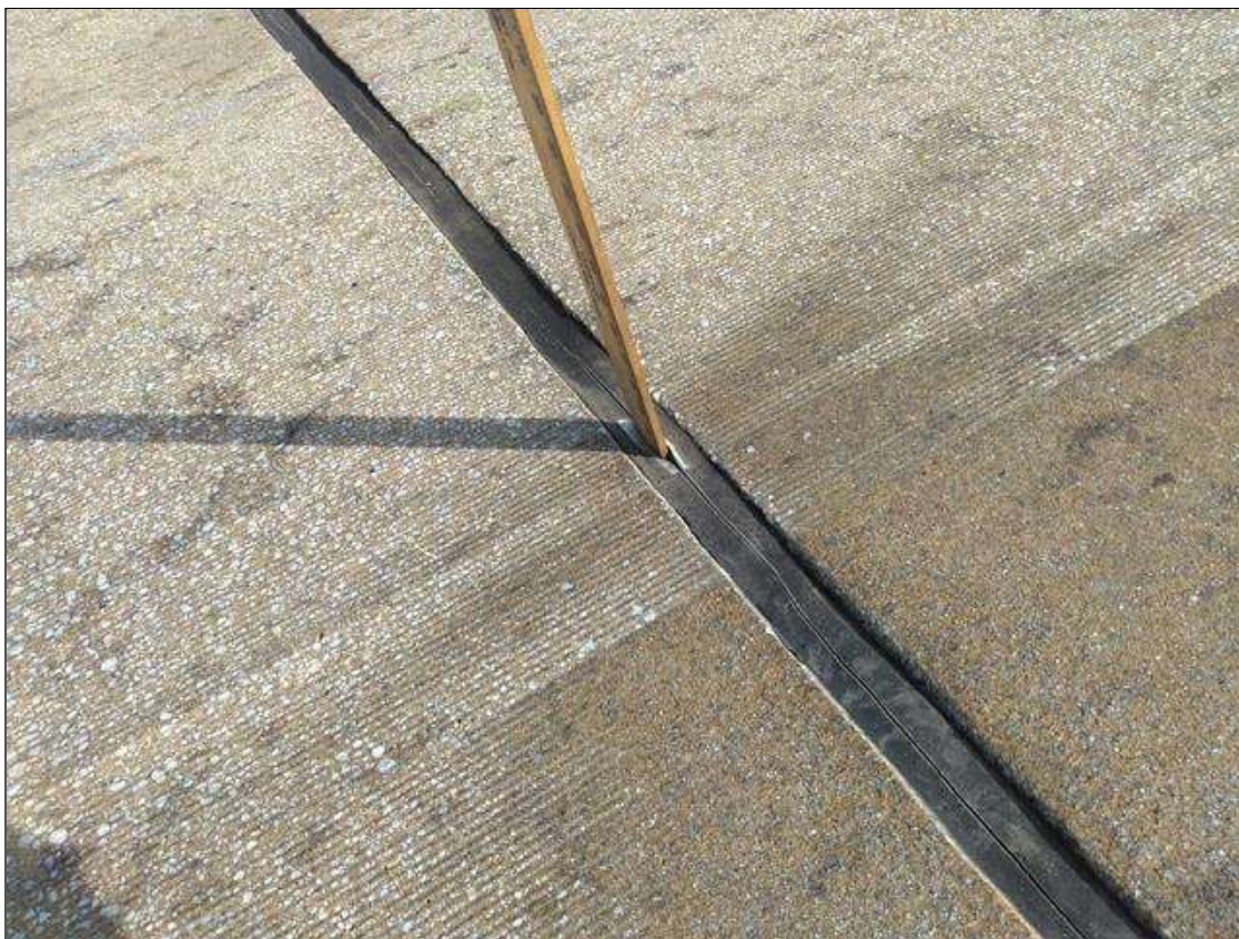
Span 221 Expansion Joint Bent 220: AT BENT 220, INTERMITTENT THROUGHOUT FULL DEPTH CRACK
