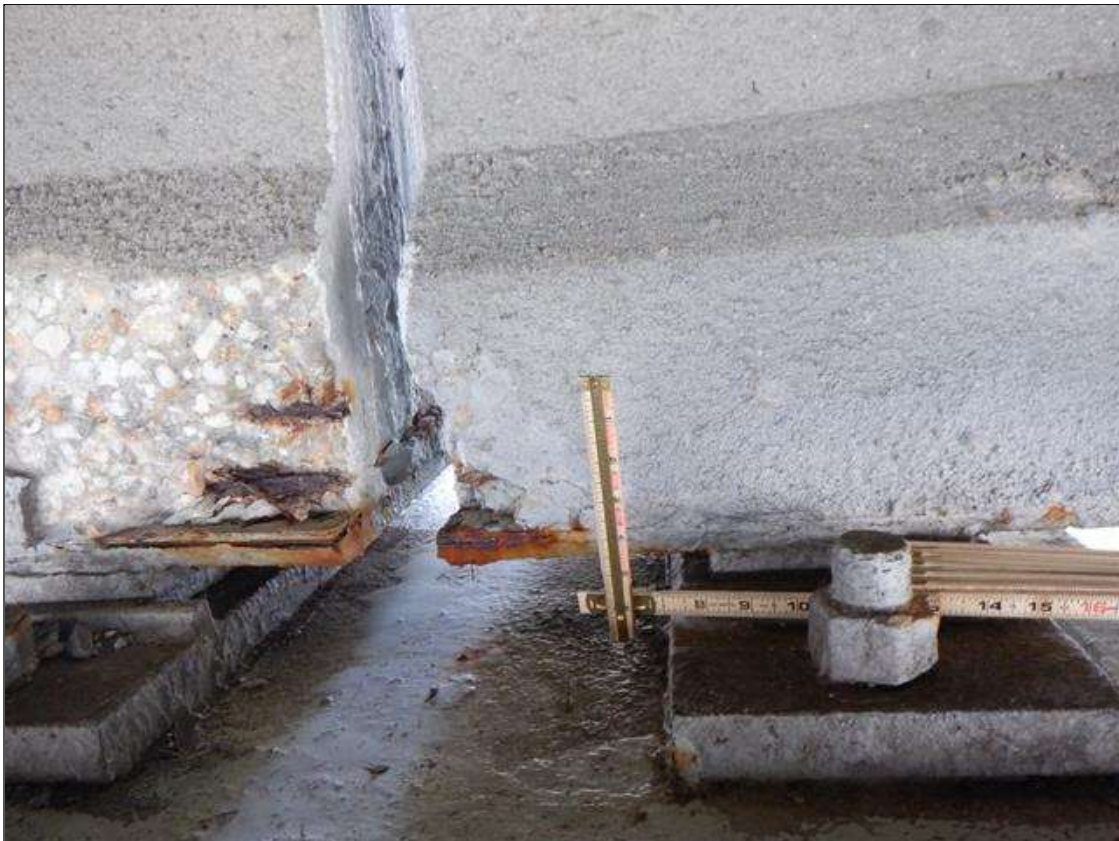
Span 110 Beam 1: (PAR) SOUTH FACE OF BOTTOM FLANGE AT BENT 109, SPALL (5 INCHES LONG X 5 INCHES HIGH X 2 INCHES DEEP) WITH (1) EXPOSED STRAND (NO LOSS)
