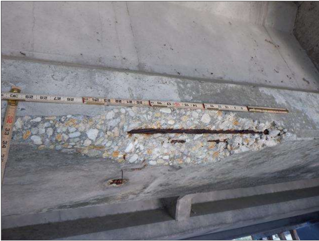
Span 221 Beam 3: (PAR) SOUTH FACE OF BOTTOM FLANGE, AT 22 FEET FROM BENT 221, SPALL (24INCHES X 8INCHES X 2 INCHES) WITH (2) EXPOSED RUSTED STRANDS (20 PERCENT SECTION LOSS) AND (1) ONE SEVERED STRAND
