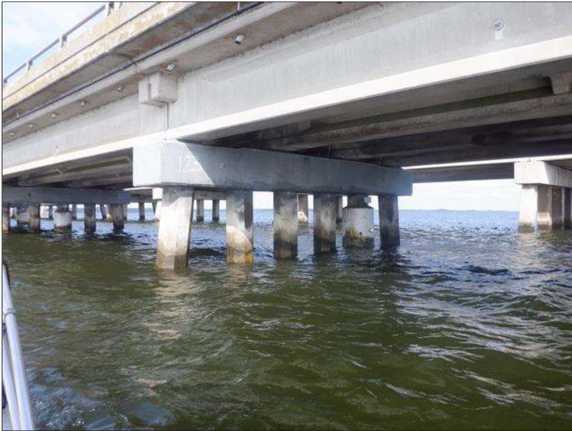
TYPICAL INTERIOR BENT PROFILE, SIX PILES IN VIEW
