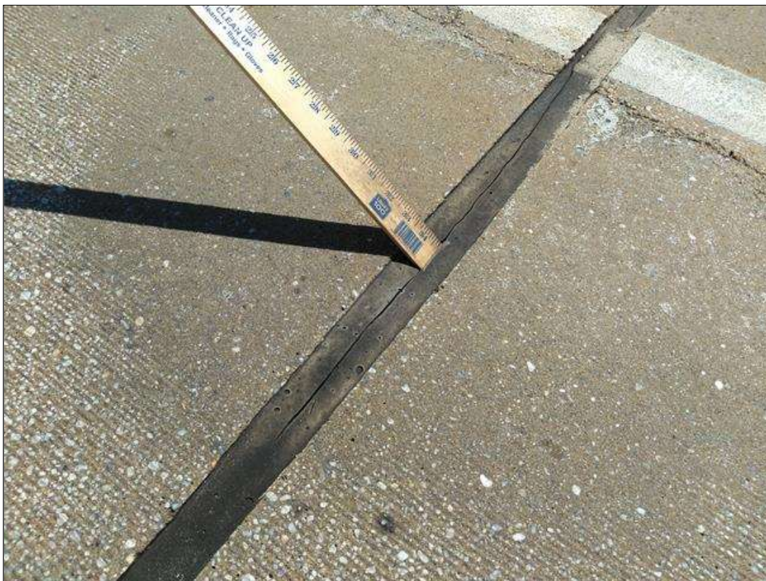
Span 56 Expansion Joint Bent 55: AT BENT 55, INTERMITTENT FULL DEPTH CRACKS THROUGHOUT
