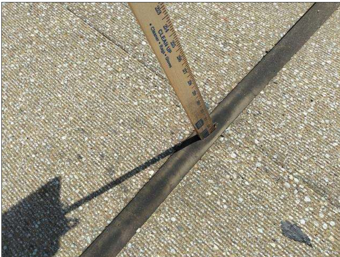
Span 41 Expansion Joint Bent 40: AT BENT 40, RIGHT LANE FULL DEPTH CRACK 2 INCHES WIDE
