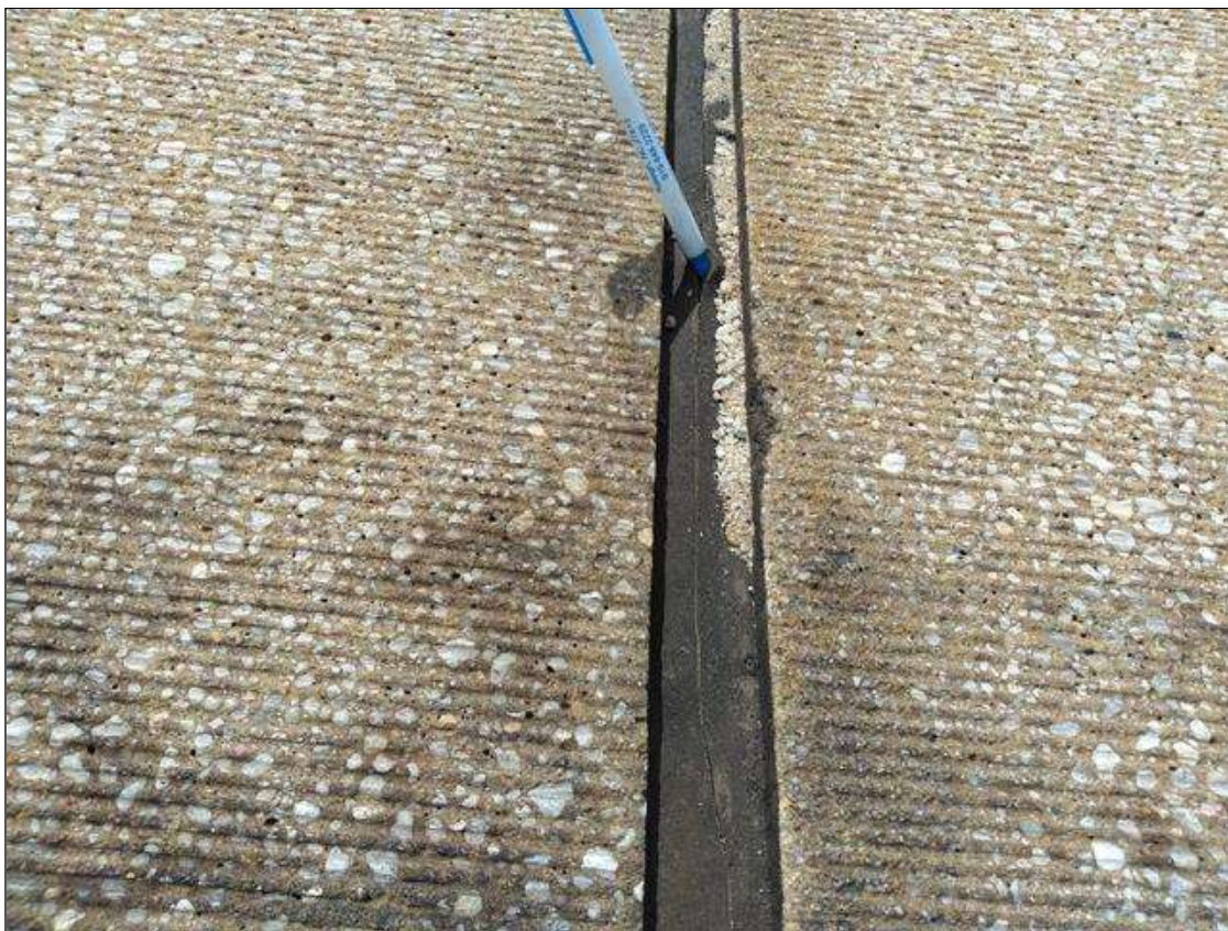
Span 248 Expansion Joint Bent 247: AT BENT 247 INTERMITTENT PARTIAL DEPTH CRACKS THROUGHOUT
