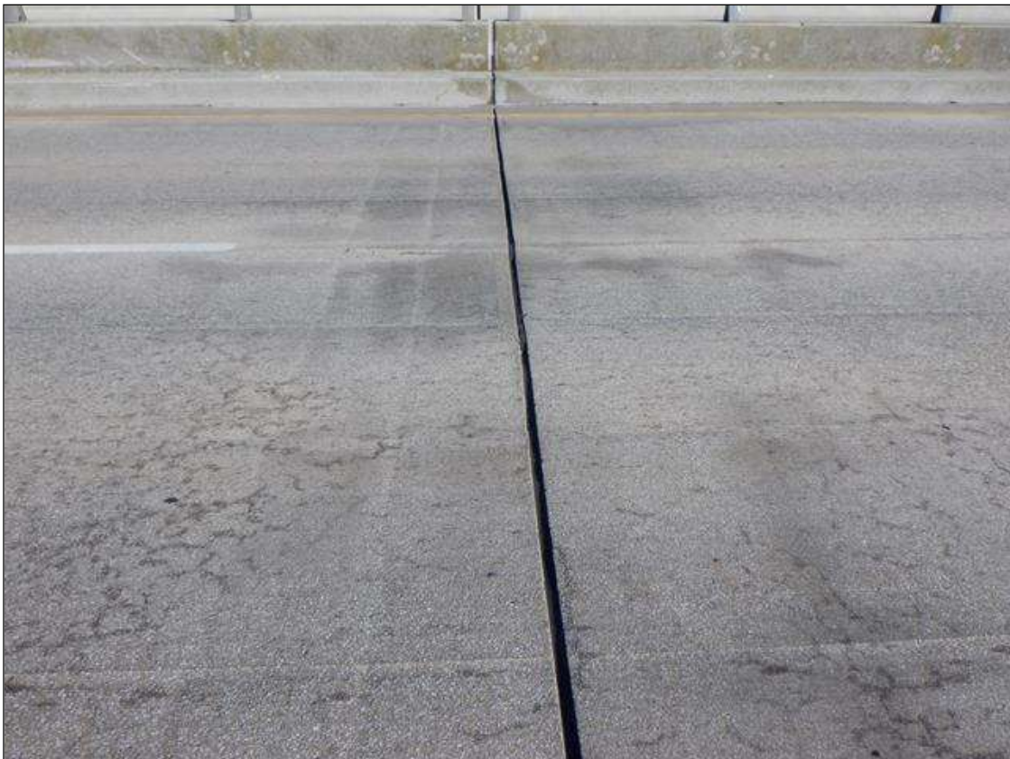
TYPICAL JOINT OVER INTERIOR BENT, JOINT OVER BENT 182 IN VIEW
