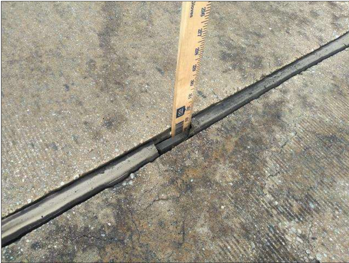
Span 103 Expansion Joint Bent 102: BOTH LANES SCATTERED THROUGHOUT, LOSS OF ADHESION (5FEET X FULL DEPTH)
