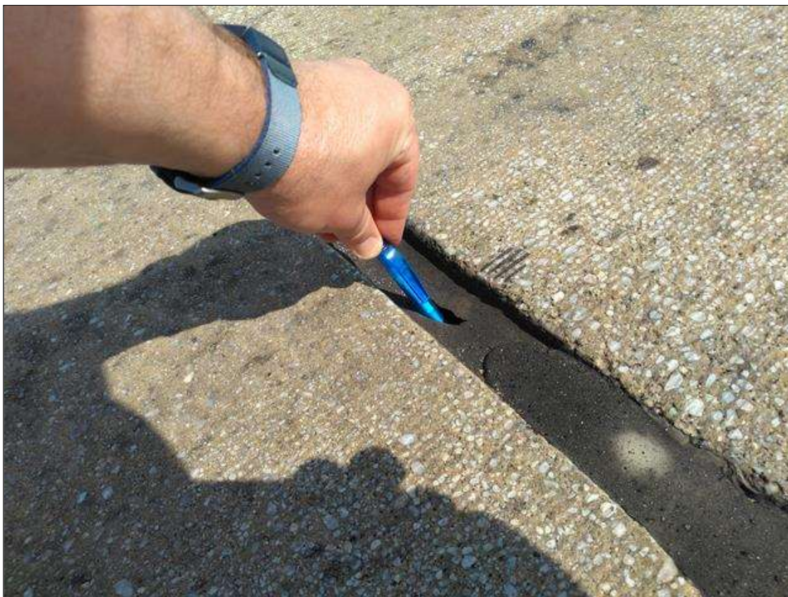
Span 141 Expansion Joint Bent 140: AT BENT 140, RIGHT LANE INTERMITTENT FULL DEPTH CRACKS UP TO 2 INCH LONG
