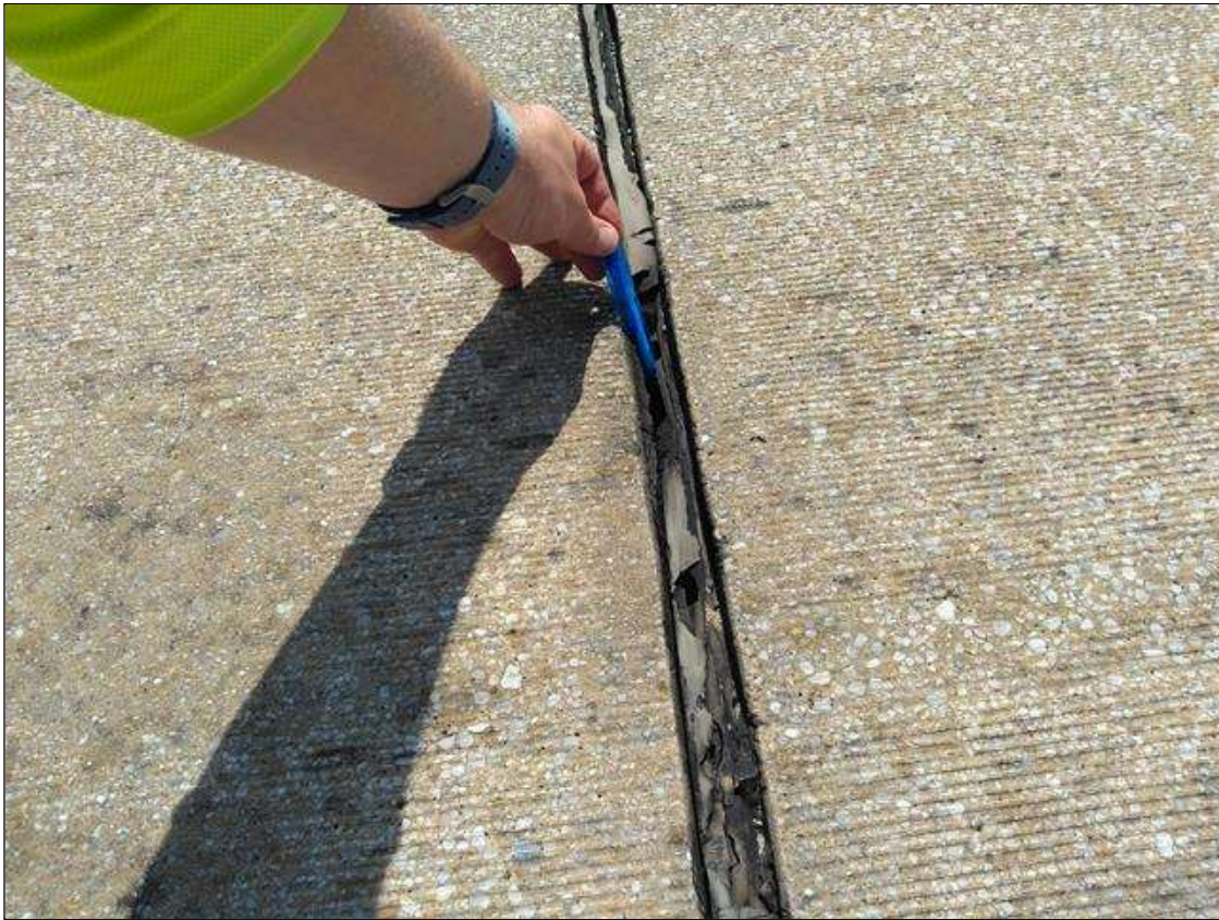
Span 170 Expansion Joint Bent 169: AT BENT 160, FULL WIDTH AND FULL DEPTH CRACKING, TORN, OR MISSING JOINT
