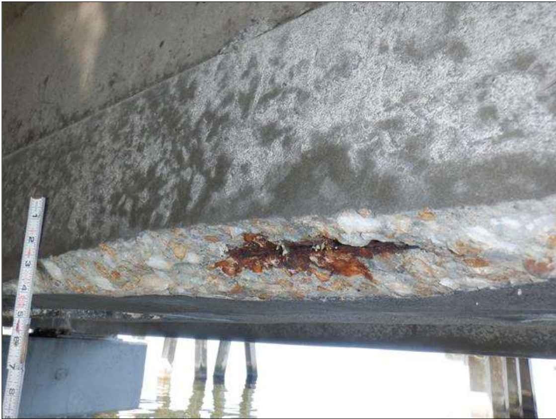
Span 157 Beam 2: (PAR) BOTTOM FLANGE ALL FACES, STARTING AT BENT 156, FAILED PATCH WITH MULTIPLE SPALLS (UP TO 2 FEET LONG X UP TO 12 INCHES WIDE X UP TO 2 INCHES DEEP) WITH EXPOSED RUSTED STRANDS (10 PERCENT SECTION LOSS)
