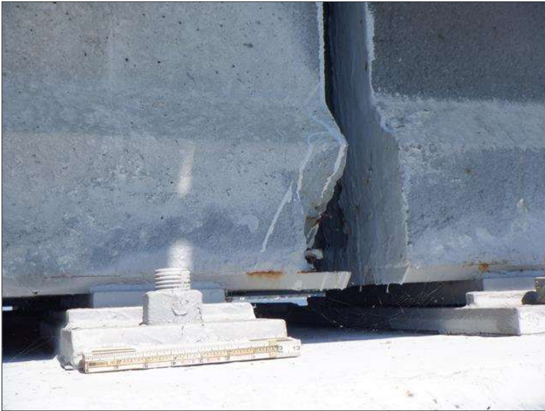
Span 225 Beam 1: (PAR) SOUTH FACE OF BOTTOM FLANGE, AT BENT 225, SPALL (7 INCHES X 8 INCHES X UP TO 3 INCHES) WITH (2) EXPOSED RUSTED STRANDS (UP TO 50 PERCENT SECTION LOSS) ON STRAND (NOT FOUND AT THIS LOCATION DURING 2022 INSPECTION)
