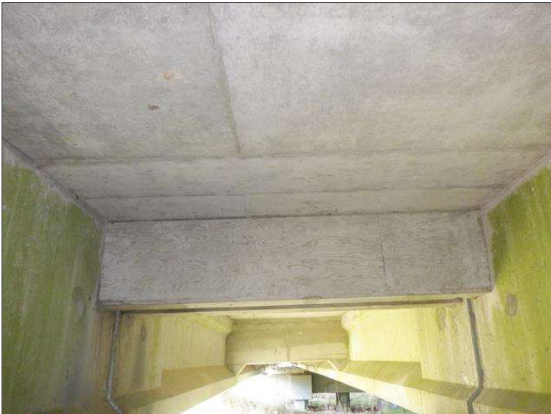
TYPICAL END DIAPHRAGM
