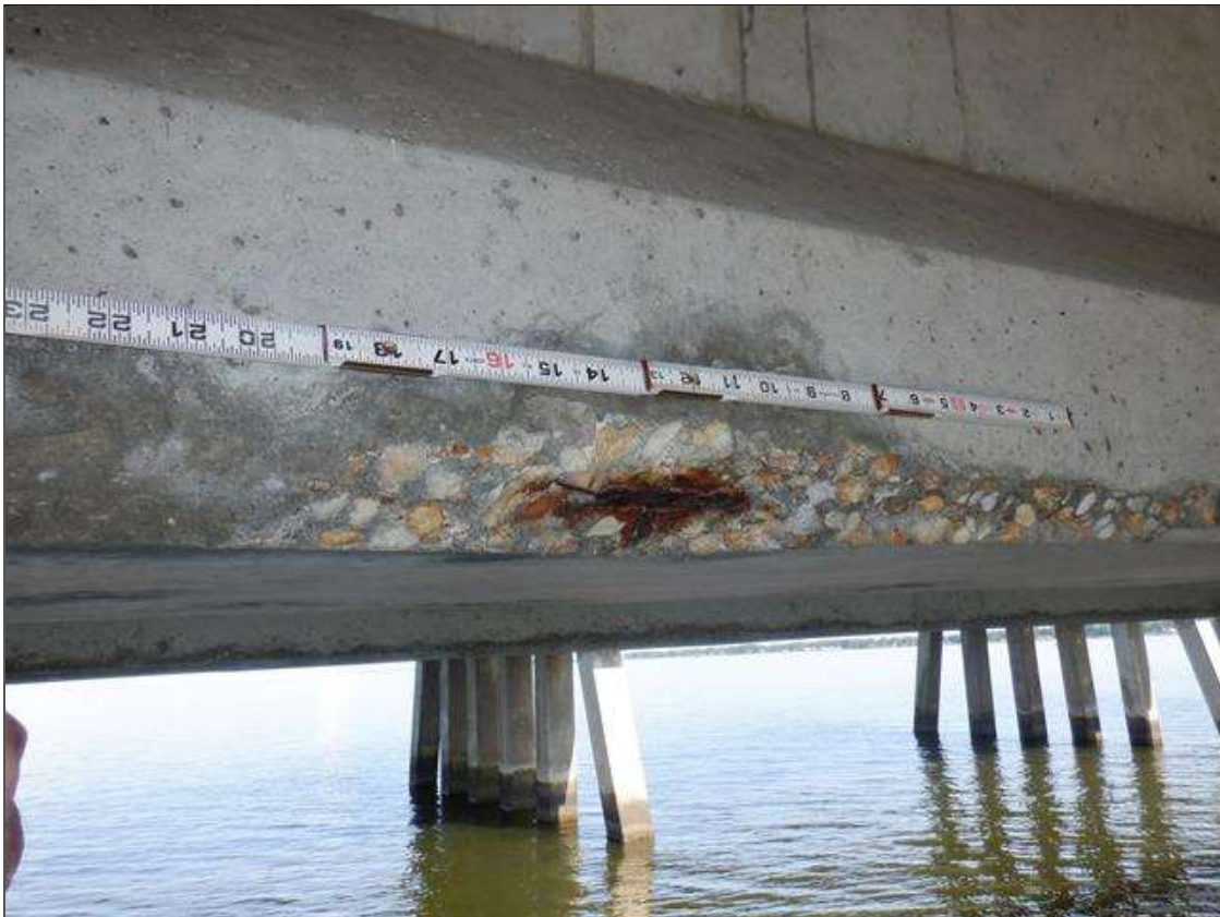
Span 161 Beam 2: (PAR) SOUTH FACE OF BOTTOM FLANGE AT MIDSPAN, SPALL (24INCHES X 4INCHES X 2 INCHES) WITH EXPOSED STRANDS (5 PERCENT SECTION LOSS) ON STRAND
