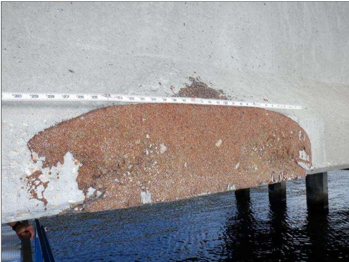
Span 3 Beam 4: SOUTH FACE OF BOTTOM FLANGE AT 25 FEET FROM BENT 2, PATCHED AREA (24 INCHES X 15 INCHES)
