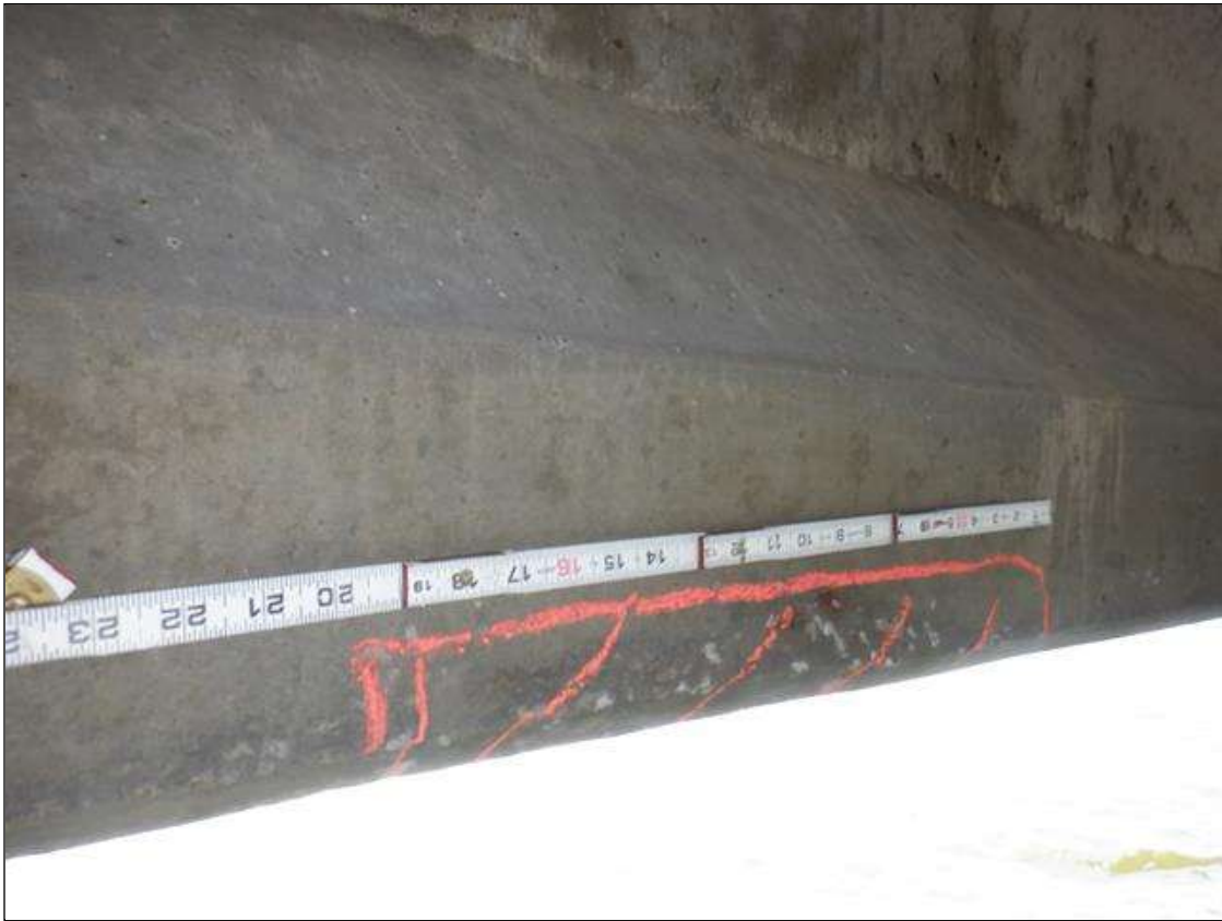
Span 37 Beam 3: BOTTOM FLANGE NORTH FACE AT 6 FEET FROM BENT 37, HORIZONTAL CRACK (UP TO 1/32 INCH) WITH RUST STAIN AND ASSOCIATED DELAMINATION (20 INCHES X 3 INCHES)
