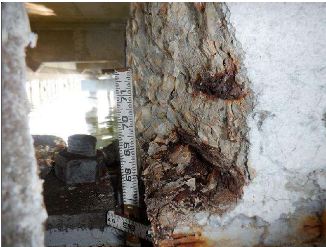
Span 156 Beam 2: (PAR) BOTTOM FLANGE NORTH FACE AT BENT 155, SPALL (15 INCHES LONG X 6 INCHES HIGH X UP TO 2 INCHES DEEP) WITH (2) TWO EXPOSED RUSTED STRANDS (10 PERCENT SECTION LOSS)
