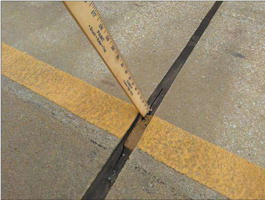
Span 78 Expansion Joint Bent 77: AT BENT 77, EDGE OF LEFT LANE FULL DEPTH CRACK 1 FOOT LONG
