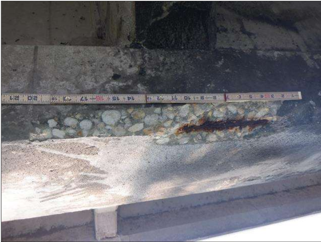
Span 223 Beam 3: (PAR) BOTTOM FLANGE NORTH FACE AT 18 FEET FROM BENT 223, SPALL (22 INCHES LONG X 2.5 INCHES HIGH X 3 INCHES WIDE X 1 INCH DEEP) WITH EXPOSED RUSTED STRANDS (10 PERCENT SECTION LOSS)
