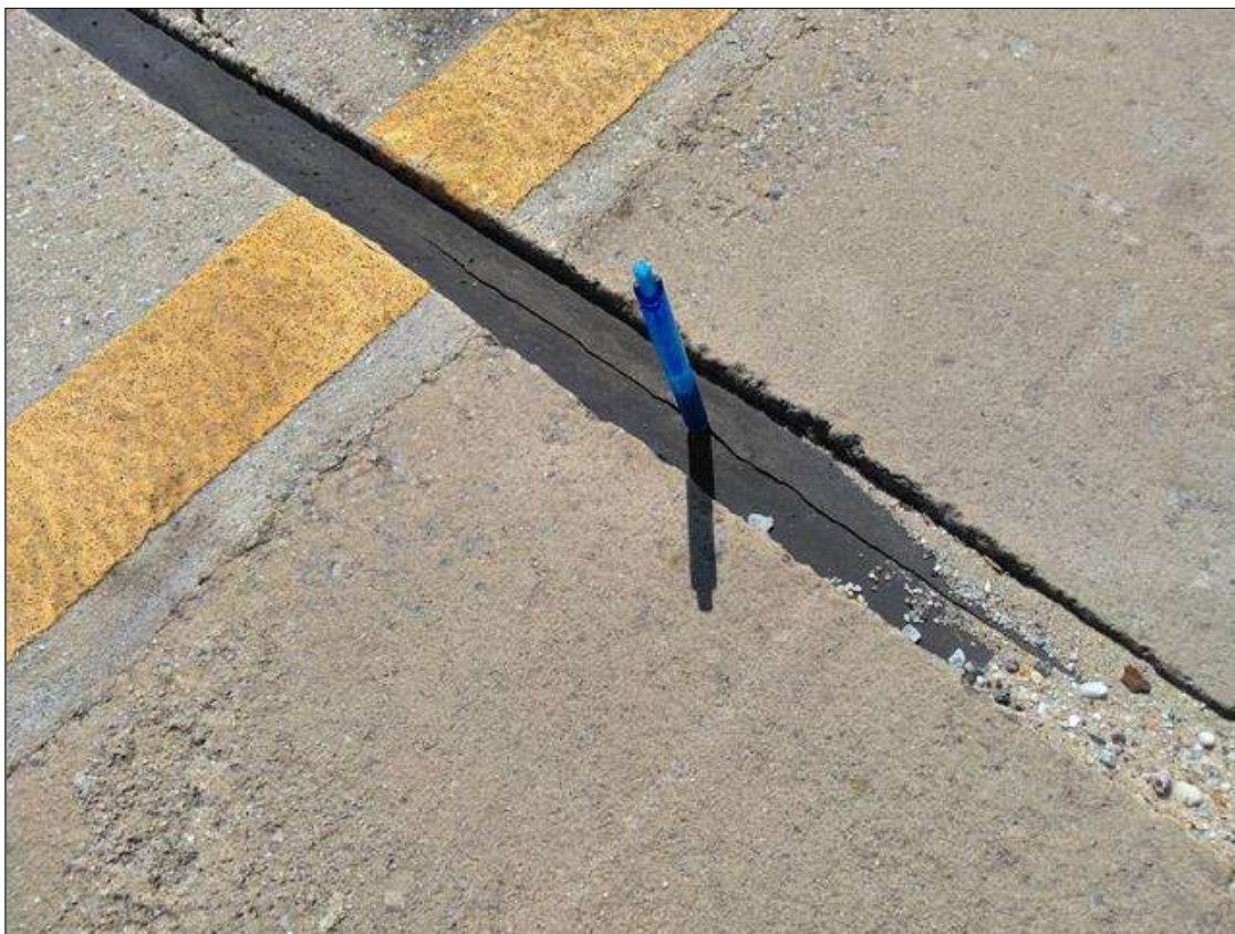
Span 178 Expansion Joint Bent 177: AT BENT 177, PARTIAL DEPTH CRACK AT LEFT SHOULDER AND CENTER
