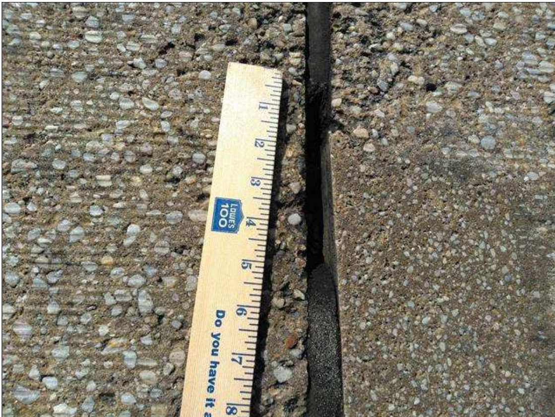
Span 23 Expansion Joint Bent 22: BENT 22 JOINT, MISSING JOINT MATERIAL LEFT LANE 5 INCH LONG PARTIAL DEPTH
