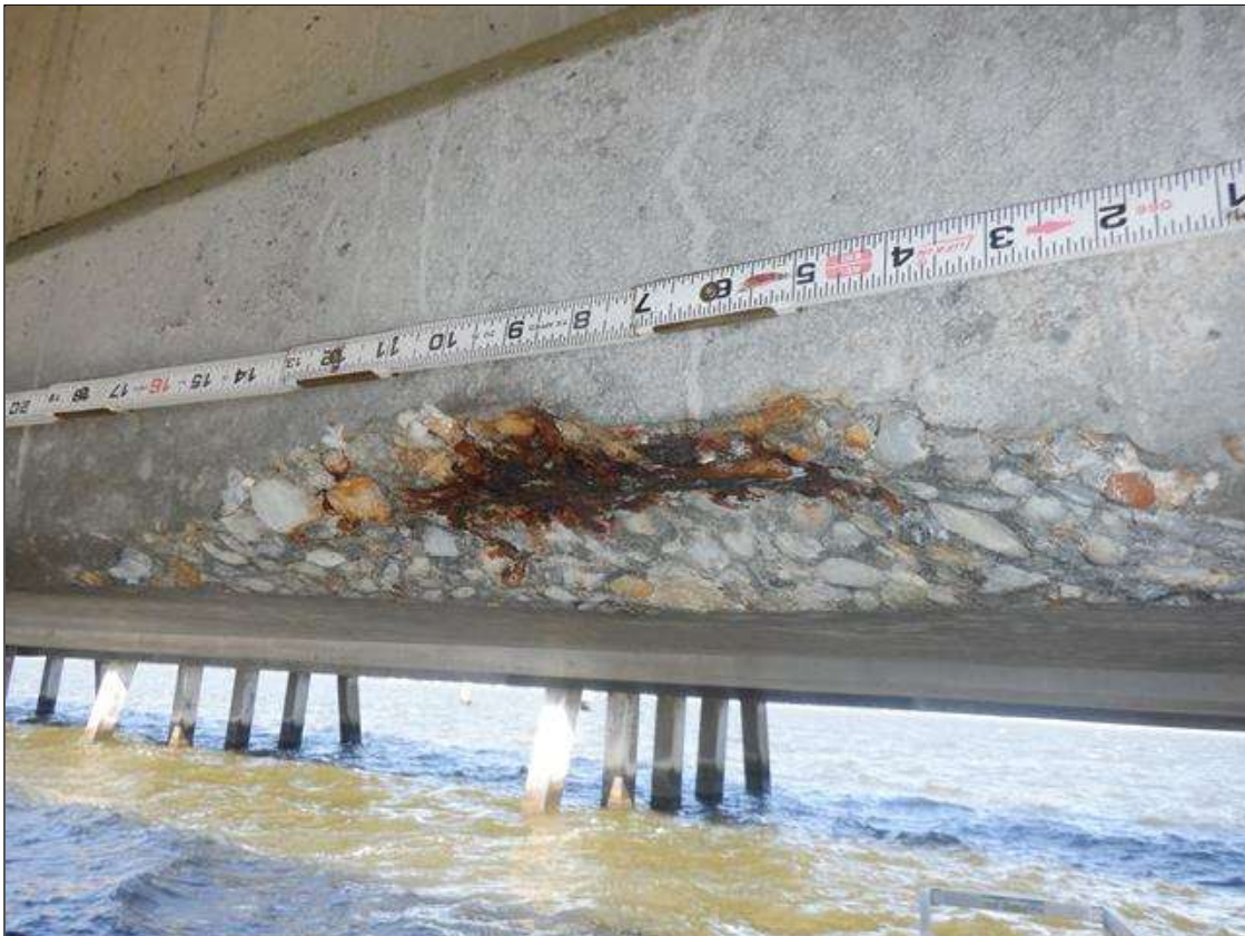
Span 100 Beam 3: (PAR) SOUTH FACE OF BOTTOM FLANGE AT 12 FEET FROM BENT 100, SPALL ( 20 INCHES X 2 INCHES X 2 INCHES DEEP) WITH 1 AREA EXPOSED RUSTED REINFORCING (10 PERCENT SECTION LOSS)
