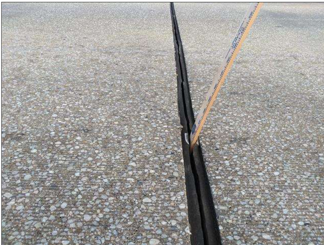
Span 13 Expansion Joint Bent 12: BOTH LANES SCATTERED THROUGHOUT, SEAL DAMAGE FULL DEPTH
