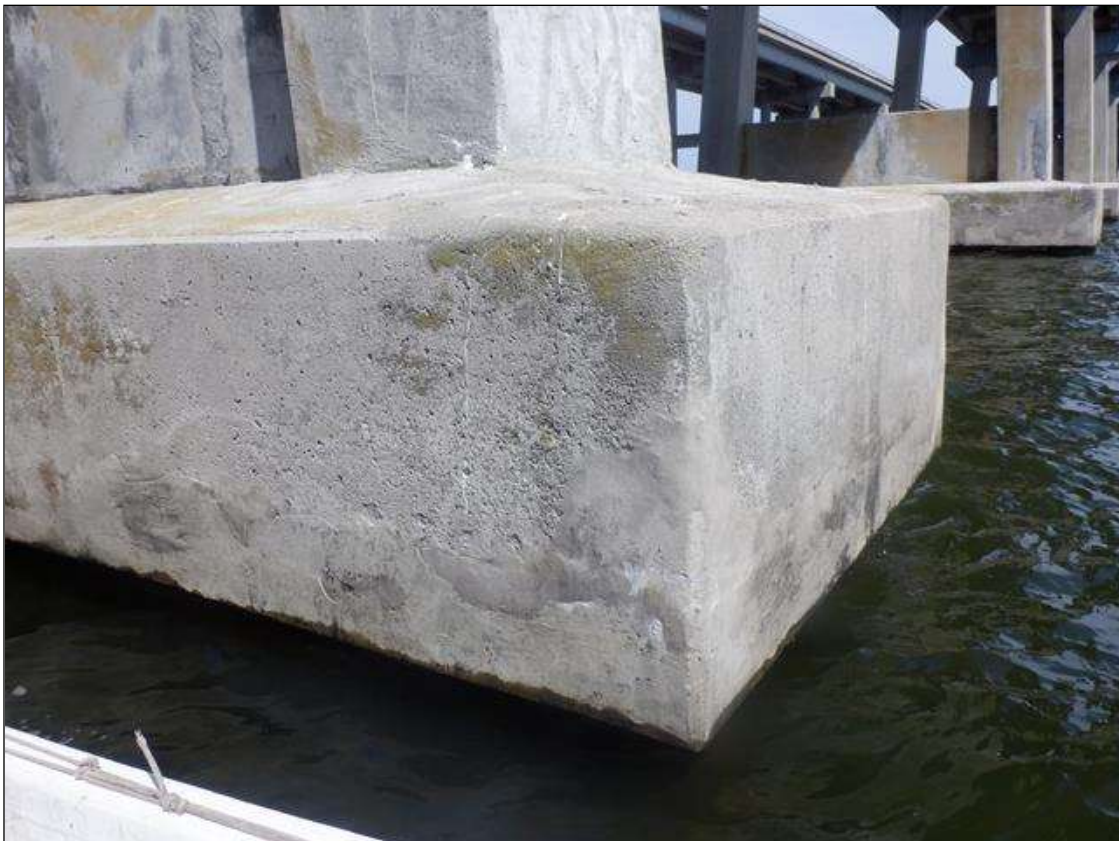
Bent 173 Footing: TOP OF WEST FACE, DELAMINATION (16FEET X UP TO 18 INCHES) SIMILAR ON EAST FACE (3FEET X 15 INCHES)
