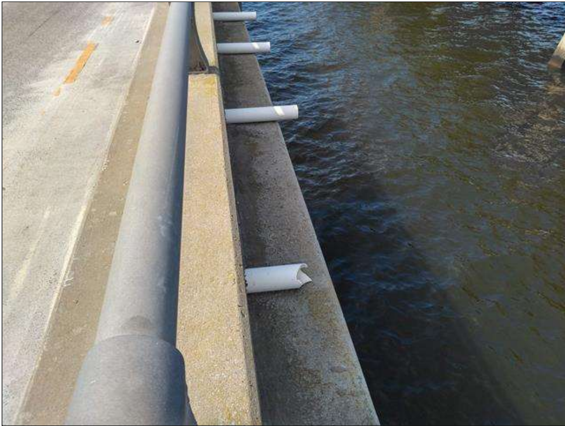
(PAR) BEHIND LEFT BARRIER ON SPAN 154 NEAR BENT 155, BROKEN SCUPPER EXTENSION PIPES
