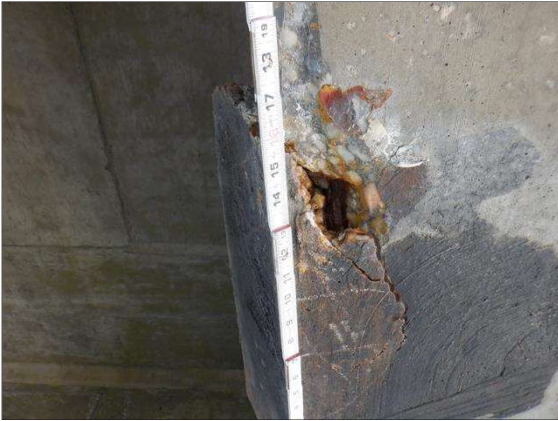
Span 203 Beam 3: (PAR) NORTH FACE OF BOTTOM FLANGE AT 13 FEET FROM BENT 202, FAILED PATCHED AREA (21 INCHES X 7 INCHES) WITH SPALL (4 INCHES X 3 INCHES X 1.5 INCHES DEEP) WITH EXPOSED RUSTED STRANDS (10 PERCENT SECTION LOSS)
