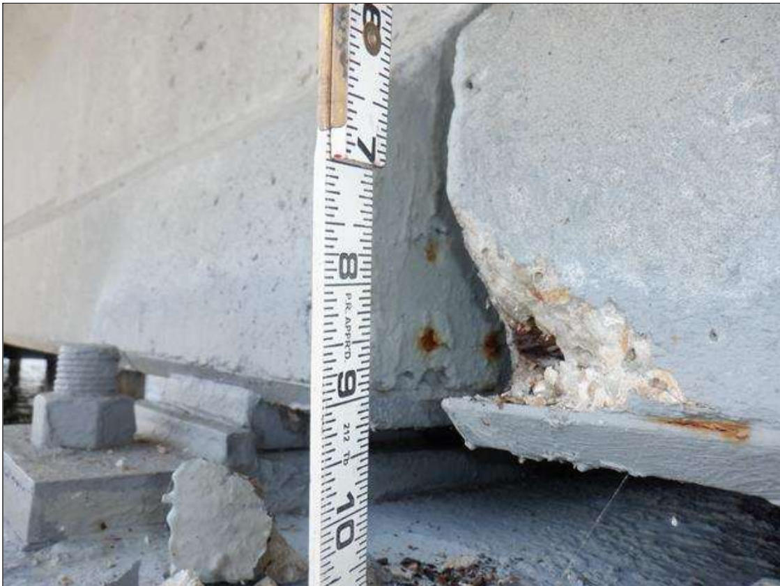
Span 42 Beam 4: BOTTOM FLANGE SOUTH FACE AT BENT 41, SPALL (3 INCHES X 3 INCHES X 2 INCHES DEEP, WITH EXPOSED RUSTED STRAND (10 PERCENT SECTION LOSS)
