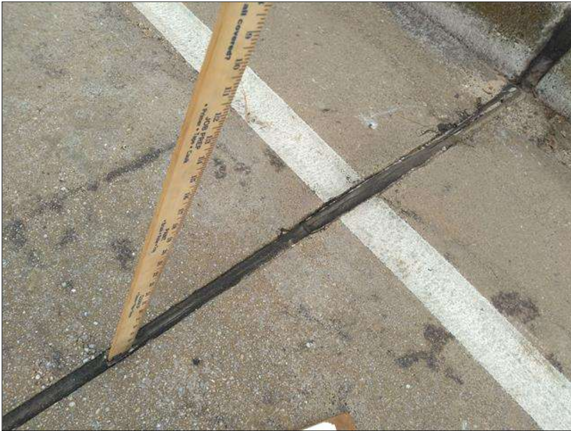
Span 100 Expansion Joint Bent 99: SCATTERED THROUGHOUT BOTH LANES, SEAL DAMAGED AND TORN (18 FEET)
