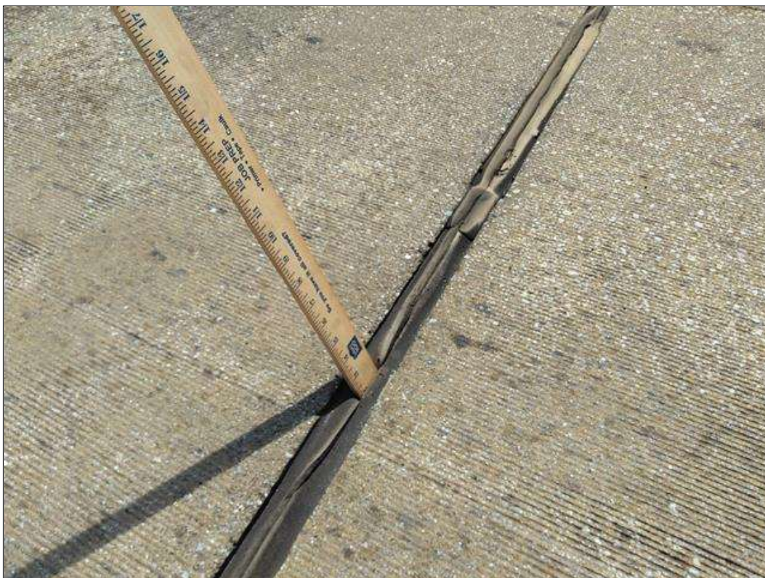
Span 43 Expansion Joint Bent 42: BOTH LANES AND SHOULDERS, SEAL DAMAGE (FULL DEPTH X FULL WIDTH)
