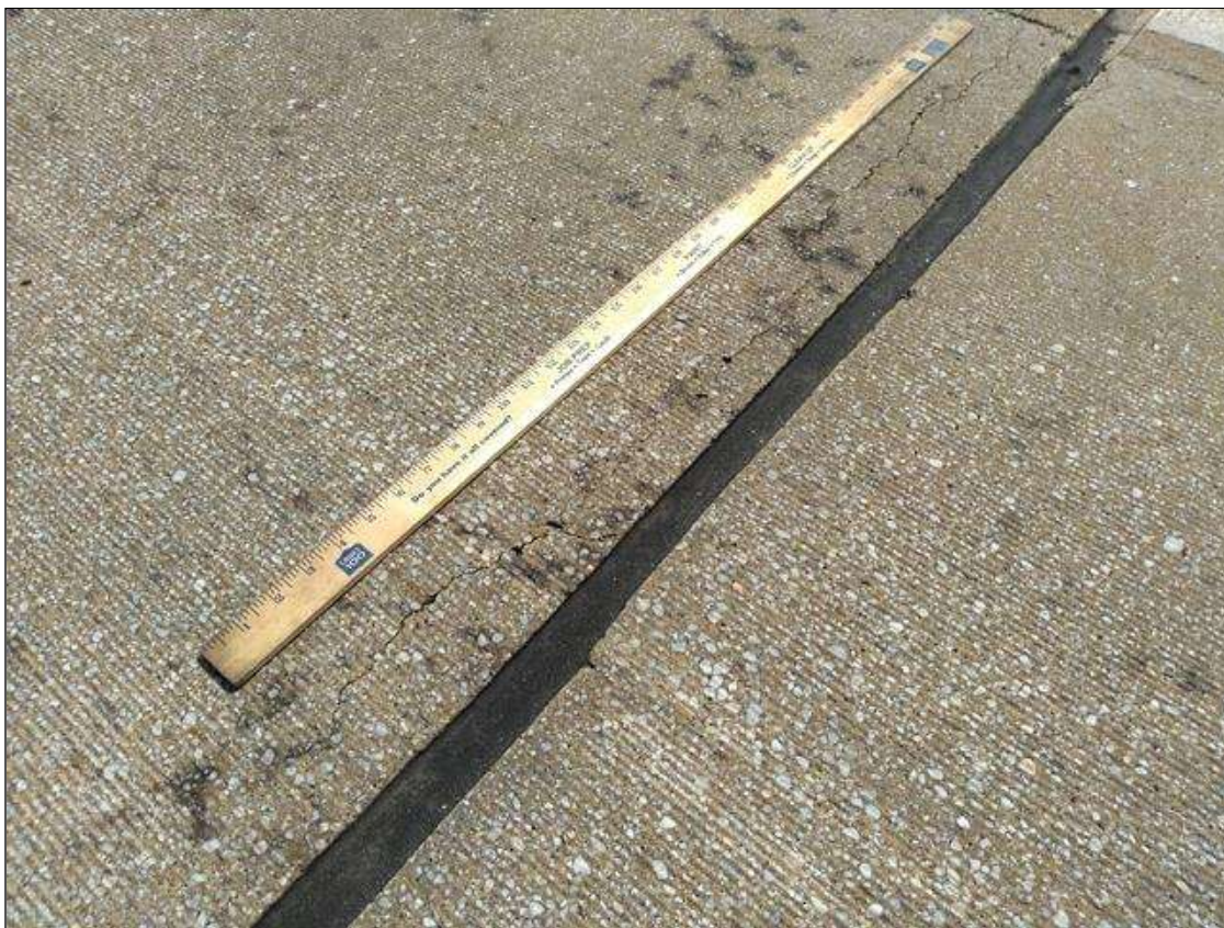
Span 163 Expansion Joint Bent 162: AT BENT 162, RIGHT LANE DELAMINATION 4 FEET WIDE X 3 INCH LONG
