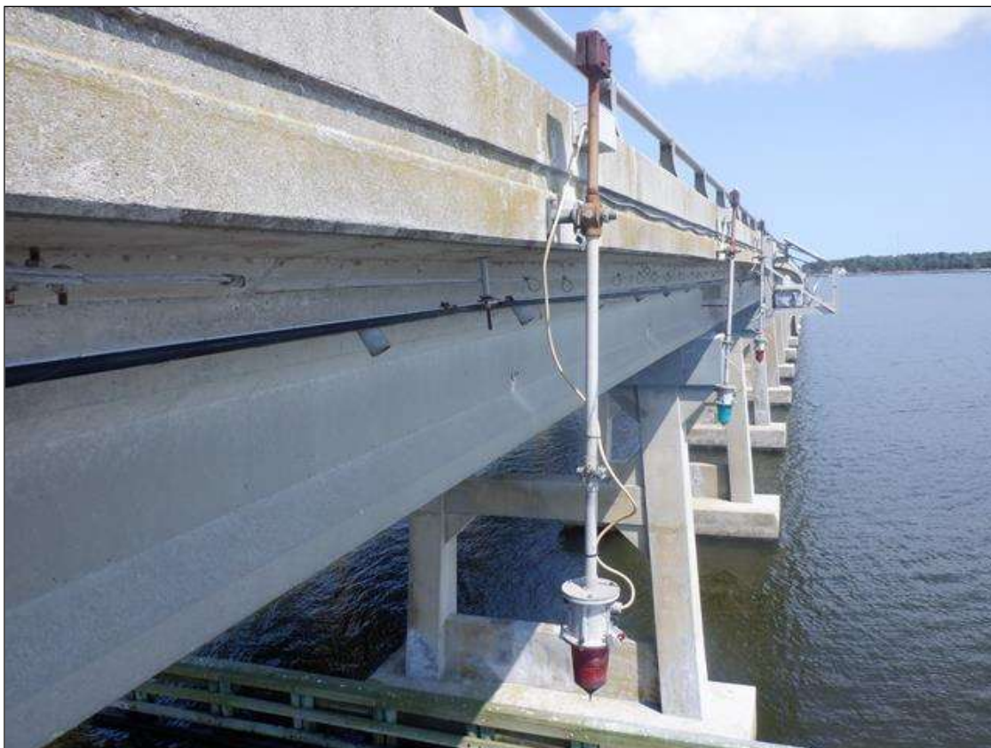
ATTACHED LIGHTING, NAVIGATIONAL AT CHANNEL
