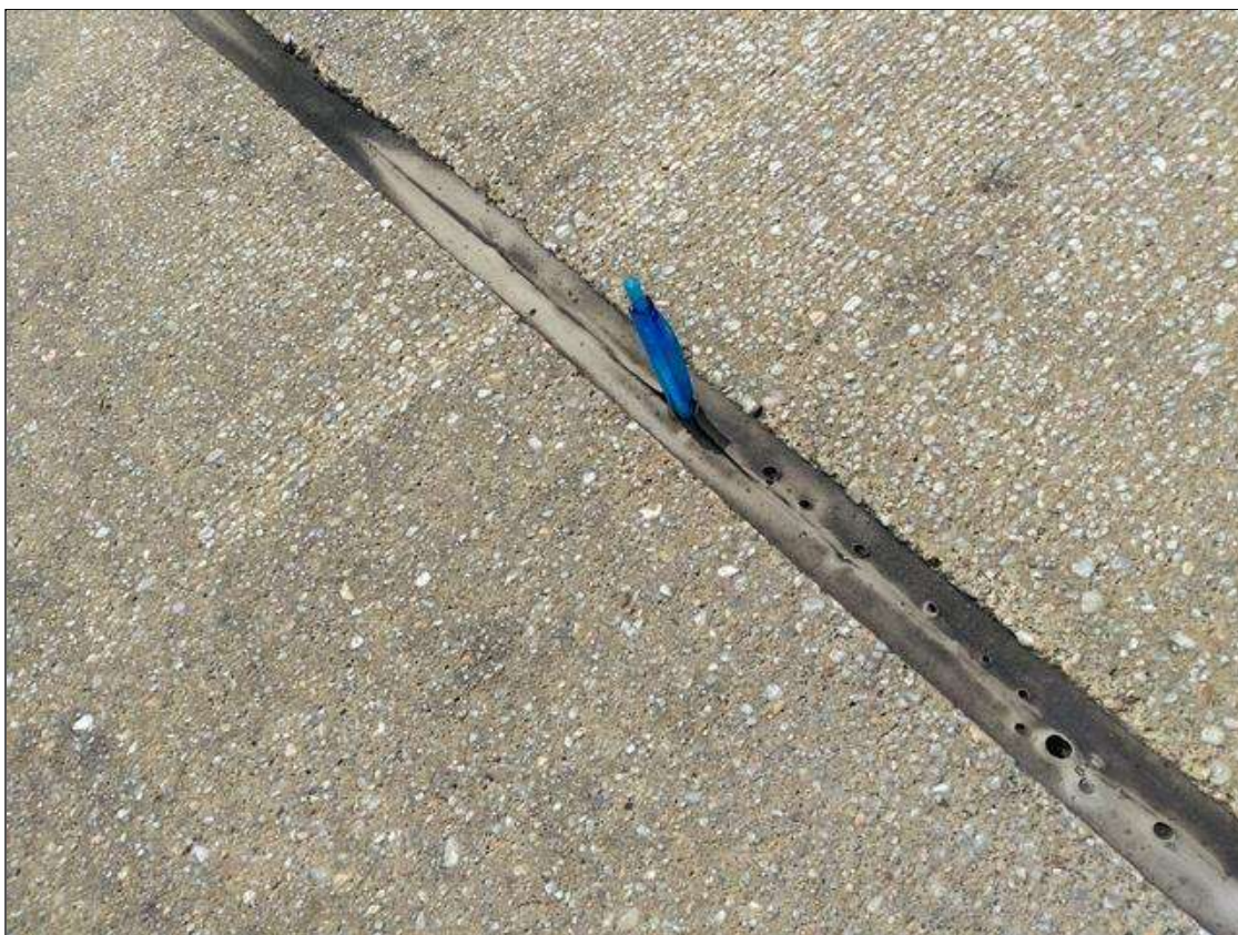
Span 158 Expansion Joint Bent 157: LEFT LANE, SEAL DAMAGE FULL DEPTH (4 FEET)
