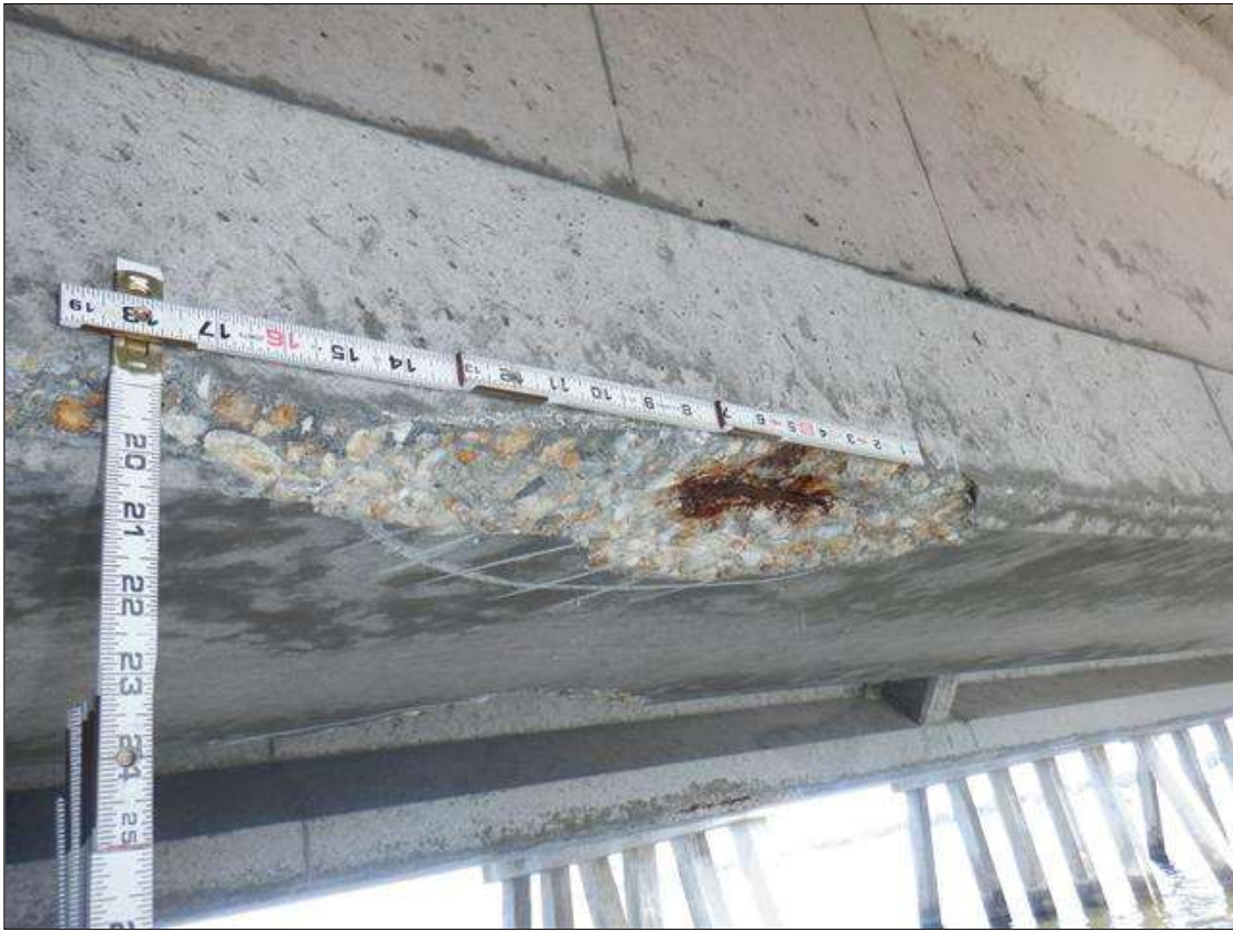
Span 163 Beam 2: (PAR) BOTTOM FLANGE, SOUTH AND BOTTOM FACES, 7 FEET FROM BENT 162, SPALL (24 INCHES X 6 INCHES X 1 INCH DEEP) WITH EXPOSED RUSTED STRANDS (10 PERCENT SECTION LOSS)
