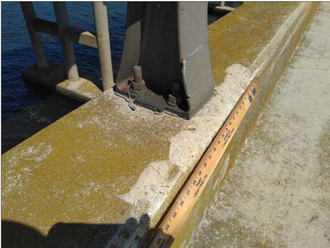
Span 175 Left Bridge Rail: AT RAIL POST 3, SPALL 24 INCH LONG X 2 INCH WIDE X 1 INCH DEEP WITH ADJACENT IMPACT DAMAGE TO POST
