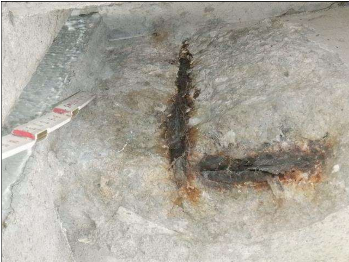
Span 21 Beam 4: END DIAPHRAGM, BAY 3 NEXT TO GIRDER 4 AT BENT 21, SPALL (12 INCHES X 15 INCHES X 2 INCHES) WITH EXPOSED RUSTED REINFORCING
