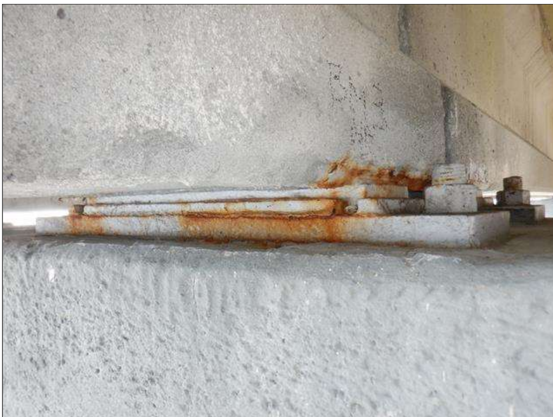
Span 15 Near Bearing: LIGHT SURFACE RUST ON BEARING
