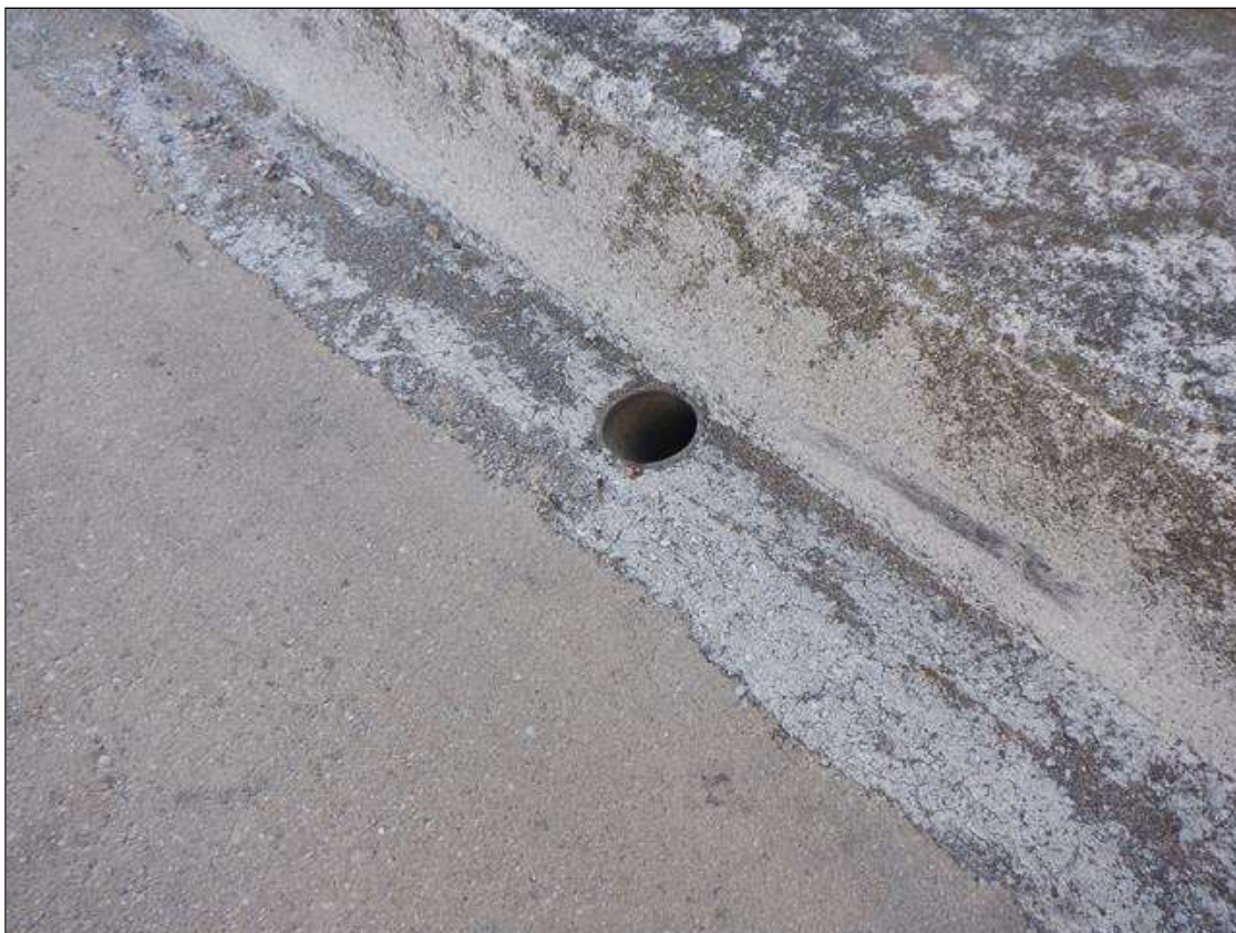
TYPICAL DECK DRAIN, TOPSIDE
