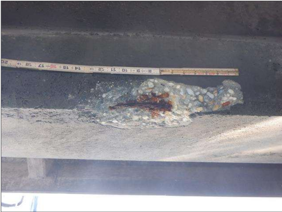
Span 215 Beam 3: (PAR) NORTH FACE OF BOTTOM FLANGE, 16 FEET FROM BENT 214, SPALL (15 INCHES X 7 INCHES X 2 INCHES DEEP X 5 INCHES OF BOTTOM FACE) WITH EXPOSED STRAND (40 PERCENT SECTION LOSS) ON STRAND AT FAILED PATCHED AREA
