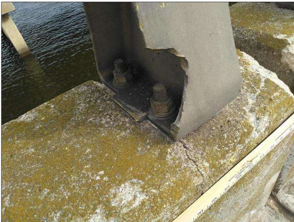
Span 5 Left Bridge Rail: RAIL POST 2, IMPACT DAMAGE (3 FEET)
