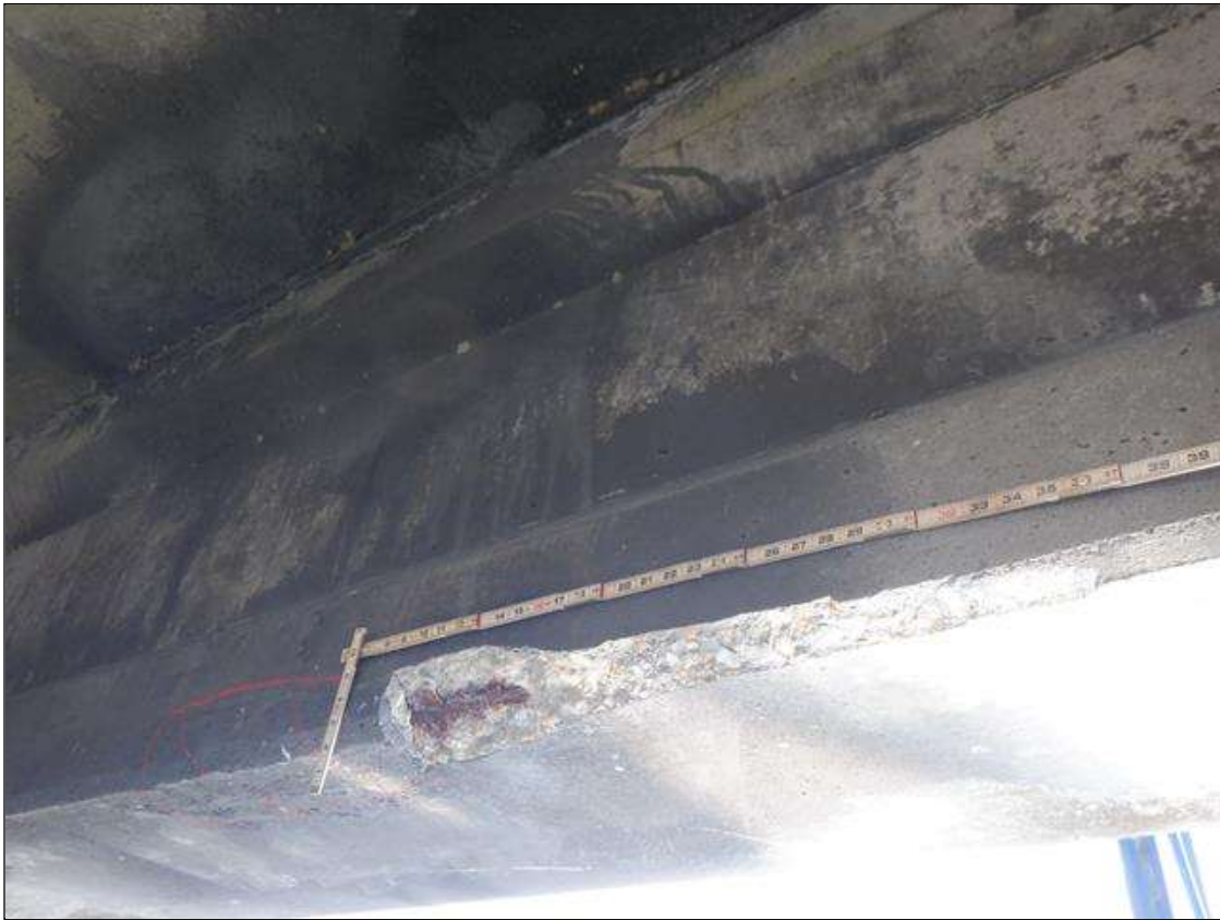
Span 131 Beam 4: (PAR) NORTH FACE OF BOTTOM FLANGE AT 12 FEET FROM BENT 131, FAILED PATCH/SPALL (44 INCHES LONG X 3 INCHES HIGH X 6 INCHES WIDE X 1.5 INCHES DEEP) WITH (1) ONE EXPOSED RUSTED STRANDS (10 PERCENT SECTION LOSS) WITH ASSOCIATED DELAMINATION (36 INCHES LONG X 5 INCHES HIGH X 7 INCHES WIDE)
