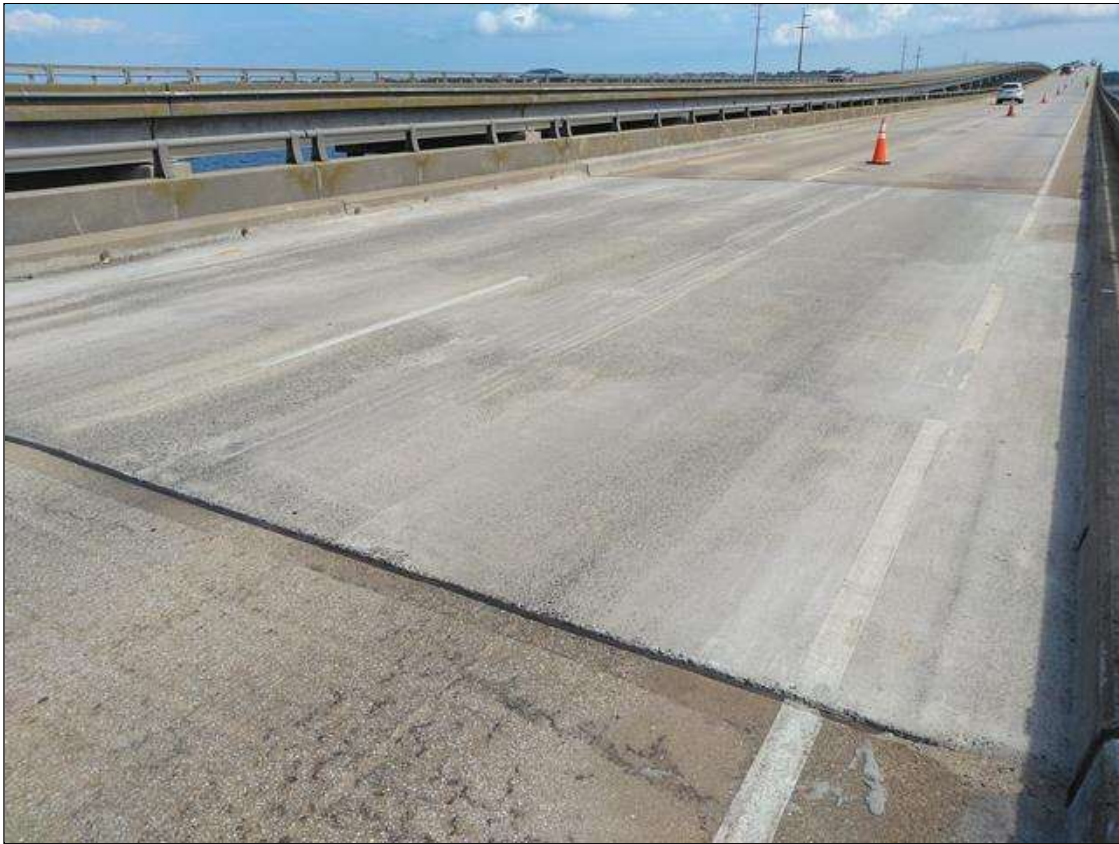
SPAN 154 CORED SLAB WITH CONCRETE WEARING SURFACE
