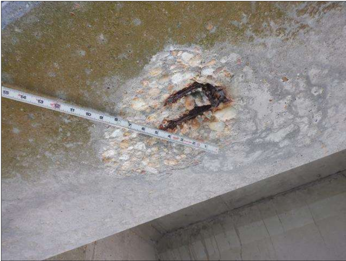
Span 185 Beam 1: (PAR) UNDERSIDE OF BOTTOM FLANGE NEAR MIDSPAN, SPALL (8 INCHES DIAMETER X 1 1/2 INCHES DEEP) WITH TWO (2) EXPOSED STRANDS (25 PERCENT LOSS)
