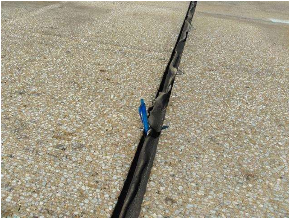
Span 192 Expansion Joint Bent 191: BENT 191, JOINT FULL WIDTH CRACKING AND TORN FULL DEPTH
