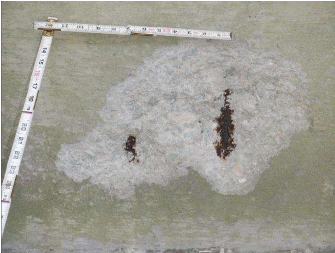
Span 51 Deck: UNDERSIDE OF DECK 5 FEET FROM BENT 51, SPALL (16 INCHES DIAMETER X 2 INCHES DEEP) WITH TWO (2) EXPOSED RUSTED REINFORCING (10 PERCENT SECTION LOSS)
