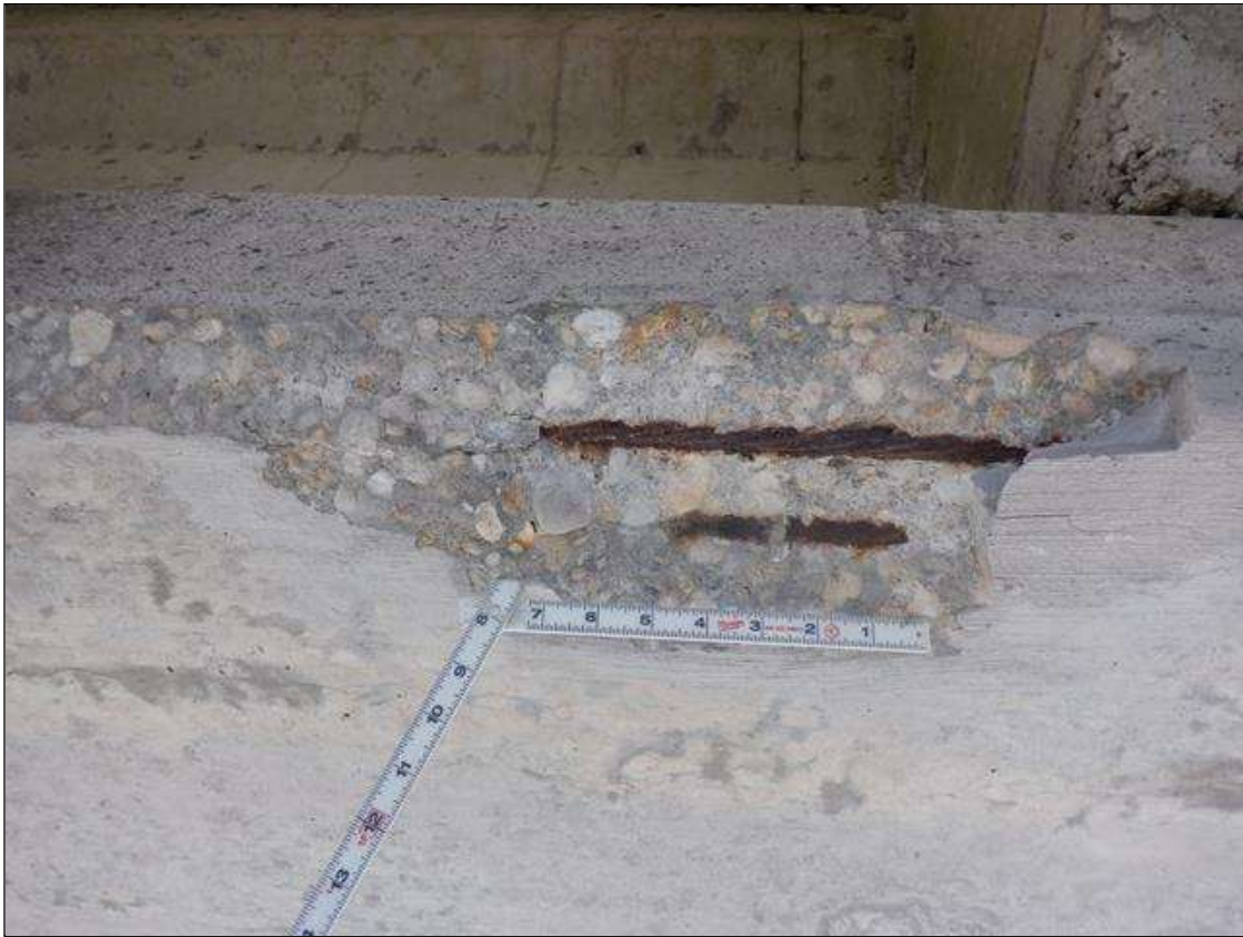
Span 178 Beam 3: (PAR) NORTH FACE OF BOTTOM FLANGE AT 21 FEET FROM BENT 177, SPALL (42 INCHES X 6 INCHES X 3 INCHES) WITH TWO (2) EXPOSED STRANDS (10 PERCENT SECTION LOSS) ON STRAND
