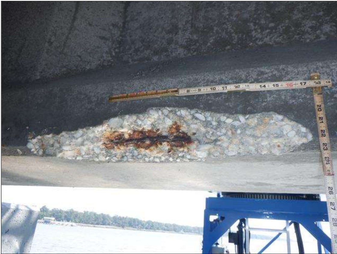
Span 230 Beam 4: (PAR) NORTH FACE OF BOTTOM FLANGE, AT 4 FEET FROM BENT 230, SPALL (24 INCHES X 6 INCHES X 2 INCHES) WITH EXPOSED RUSTED STRAND (20 PERCENT SECTION LOSS)
