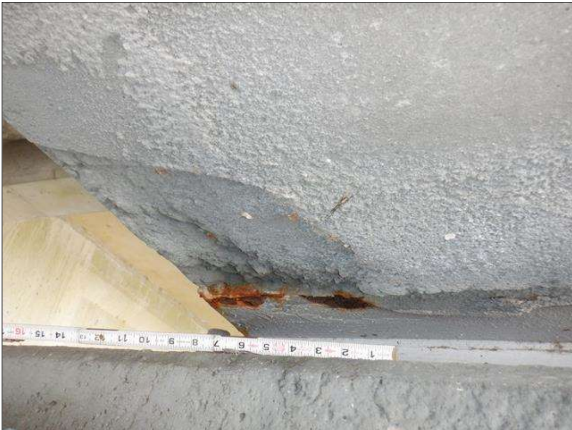
Span 4 Beam 2: 9 INCHES X 9 INCHES X 1 INCHES DEEP SPALL INCHES BOTTOM FLANGE AT PIER 4
