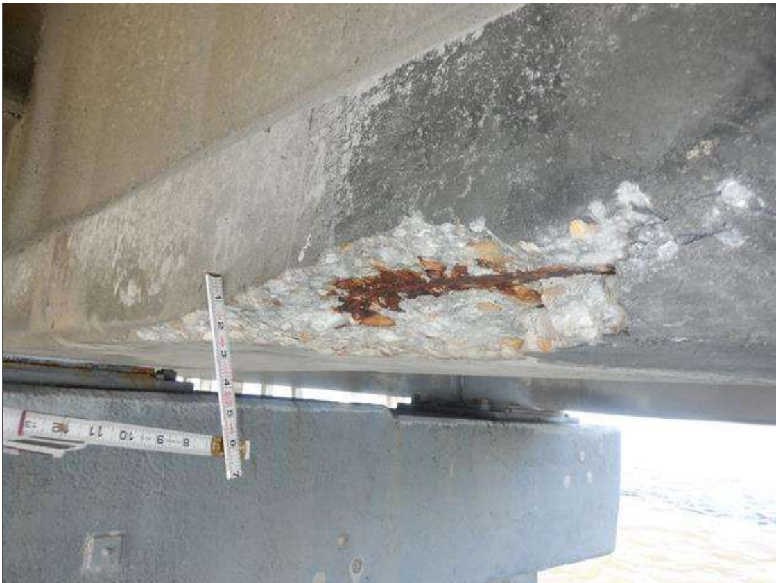
Span 100 Beam 2: (PAR) STARTING 5 FEET FROM BENT 99, SPALL/DELAMINATION (8 FEET X UP TO 9 INCHES X UP TO 2 INCHES DEEP) WITH DEBONDED STRAND
