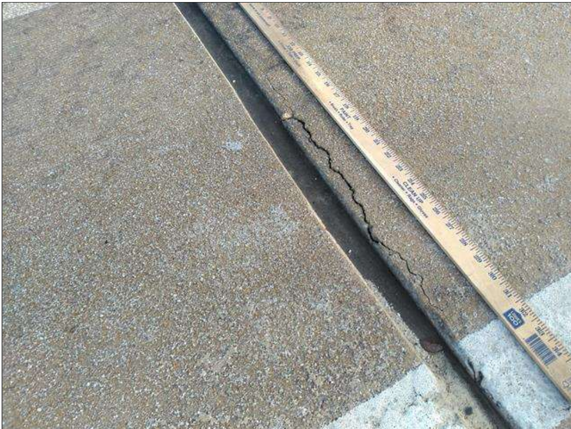
Span 206 Expansion Joint Bent 205: AT BENT 205, DELAMINATIONS AND EDGE SPALL AT RIGHT SHOULDER AND LANE. EACH 2 FEET LONG X 4 INCH WIDE X 1 INCH DEEP
