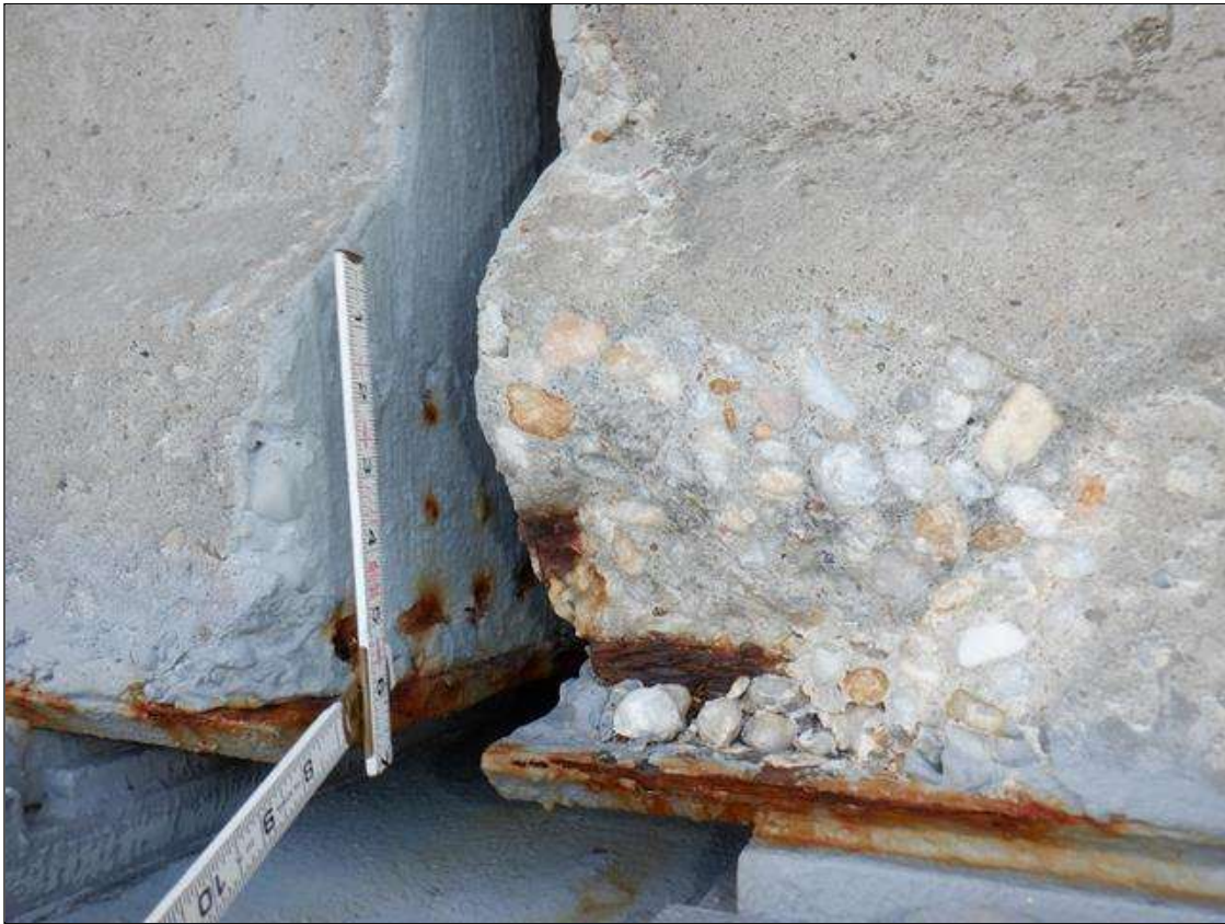
Span 52 Beam 1: (PAR) NORTH FACE OF BOTTOM FLANGE AT BENT 52, SPALL (6INCHES X 5INCHES X UP TO : 1/2INCH) WITH (2) EXPOSED RUSTED STRANDS (10 PERCENT SECTION LOSS)
