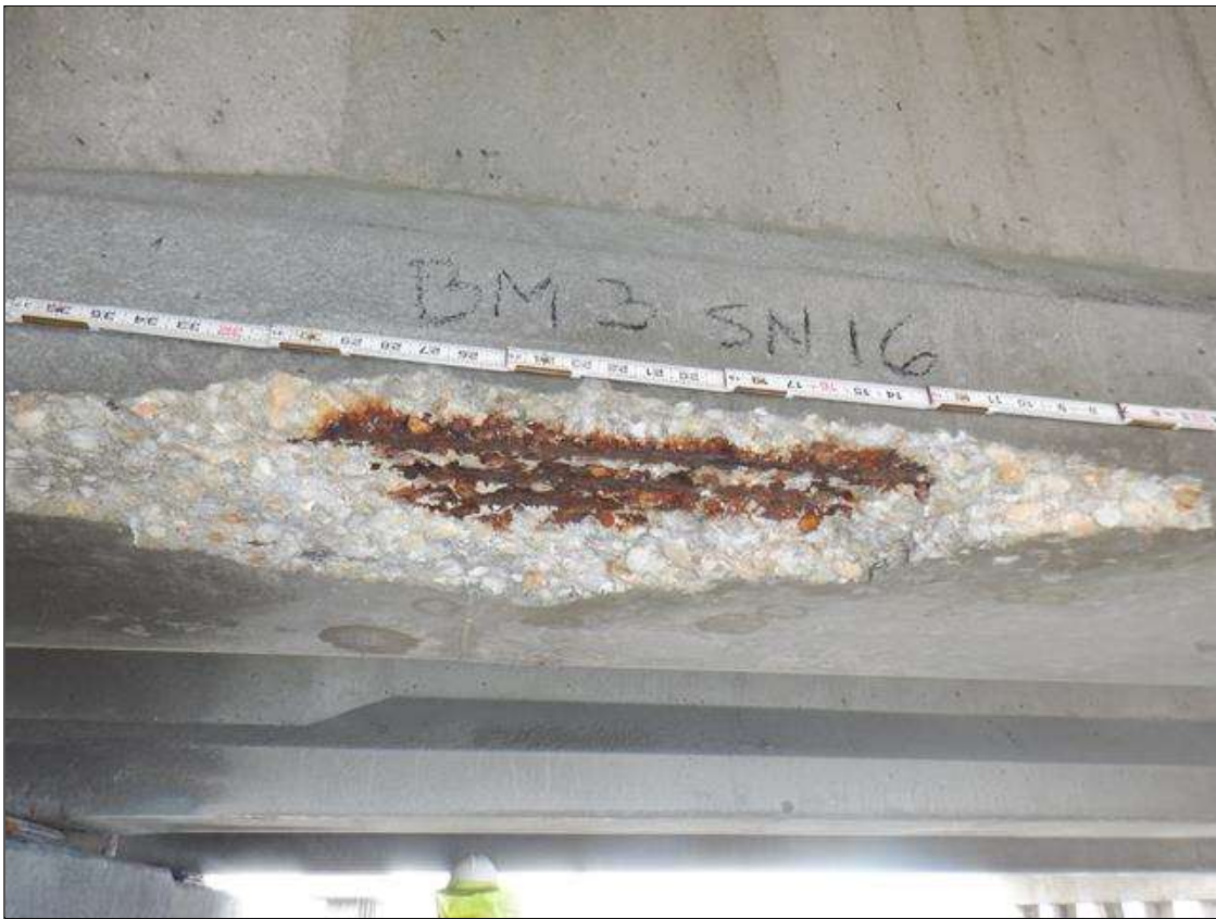
Span 16 Beam 3: (PAR) BOTTOM FLANGE SOUTH FACE, AT BENT 15, SPALL ( 4 FEET X UP TO 12 INCHES X 2 INCHES DEEP) WITH MULTIPLE EXPOSED RUSTED STRANDS (20 PERCENT SECTION LOSS)
