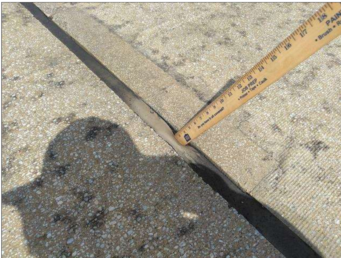
Span 63 Expansion Joint Bent 62: LEFT LANE, (2) PATCHED AREAS (UP TO 6FEET 4INCHES). NO ADHESION AT PATCHES
