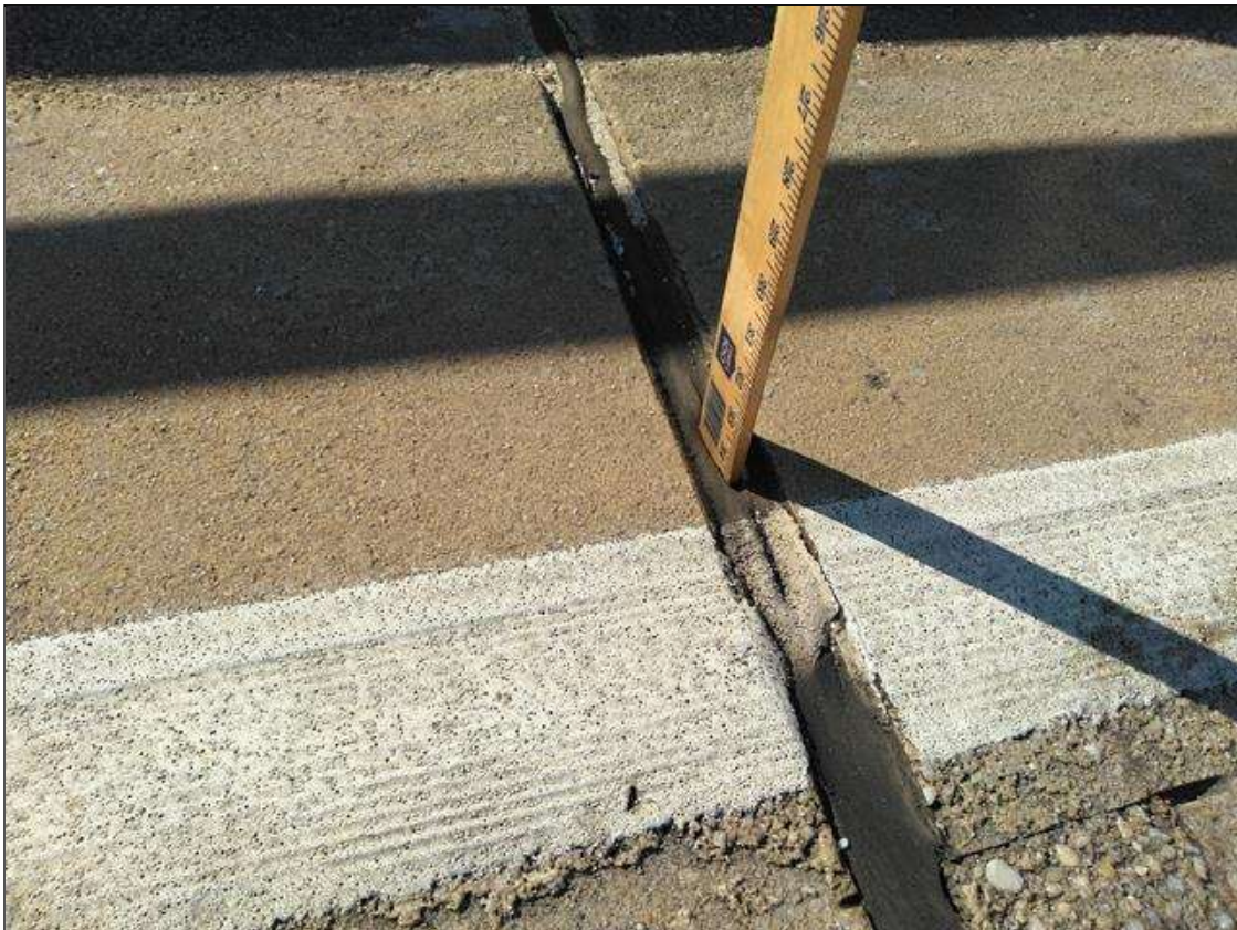
Span 214 Expansion Joint Bent 213: AT BENT 213, PARTIAL DEPTH CRACKING IN RIGHT LANE AND SHOULDER
