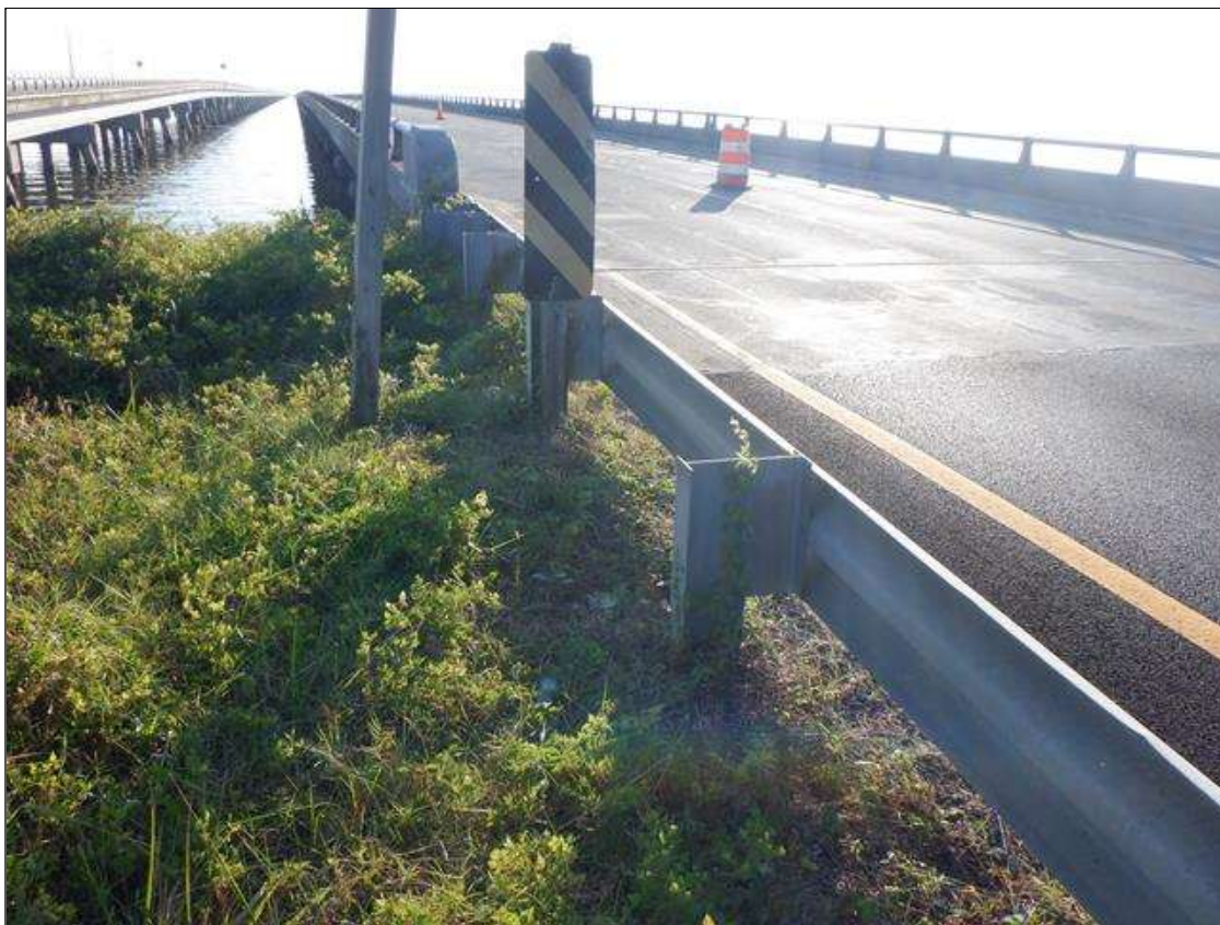
TYPICAL GUARDRAIL TRANSITION POST SPACING
