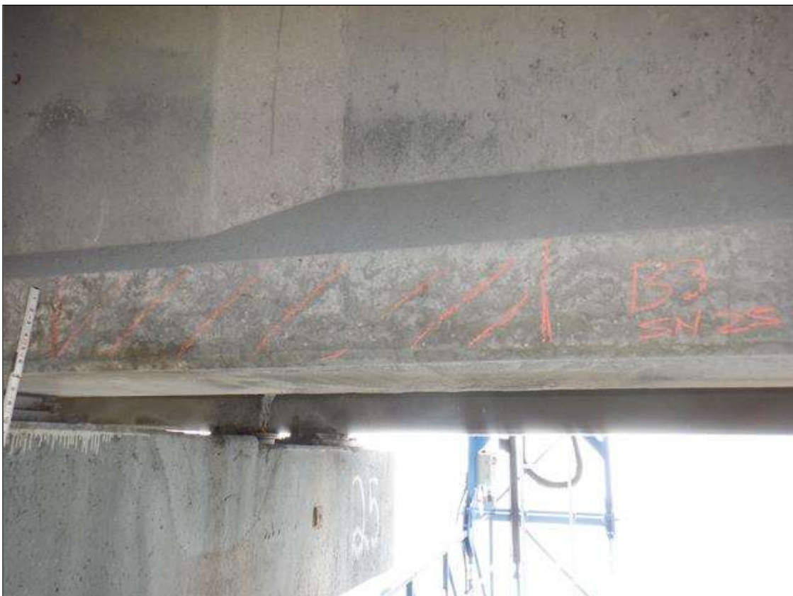
Span 25 Beam 3: BOTTOM FLANGE NORTH FACE AT BENT 25, DELAMINATION (36 INCHES X 7 INCHES)
