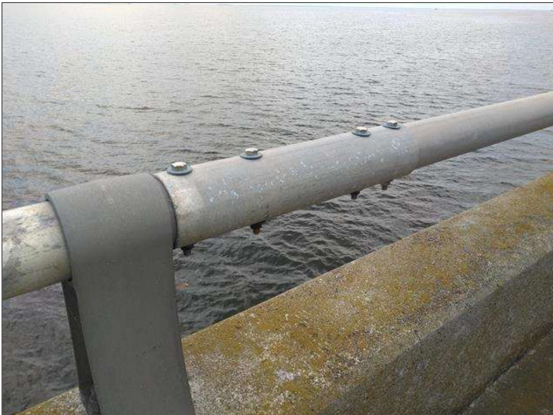
Span 70 Right Bridge Rail: METAL RAIL AT RAILPOSTS 6 AND 7, REPAIRED
