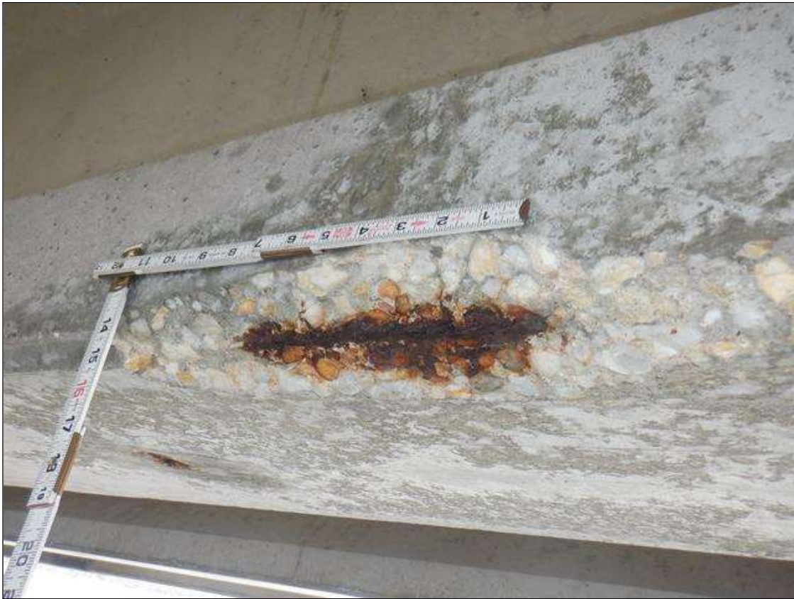
Span 205 Beam 2: (PAR) NORTH FACE OF BOTTOM FLANGE, AT 22FEET FROM BENT 204, SPALL (24INCHES X 5INCHES X 2 INCHES) WITH EXPOSED STRANDS (10 PERCENT SECTION LOSS) ON STRAND
