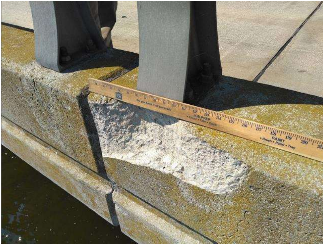
Span 195 Right Bridge Rail: AT FIRST RAIL POST (OUTSIDE) SPALL 16 INCH X 7 INCHES HIGH X 1.5 INCHES DEEP
