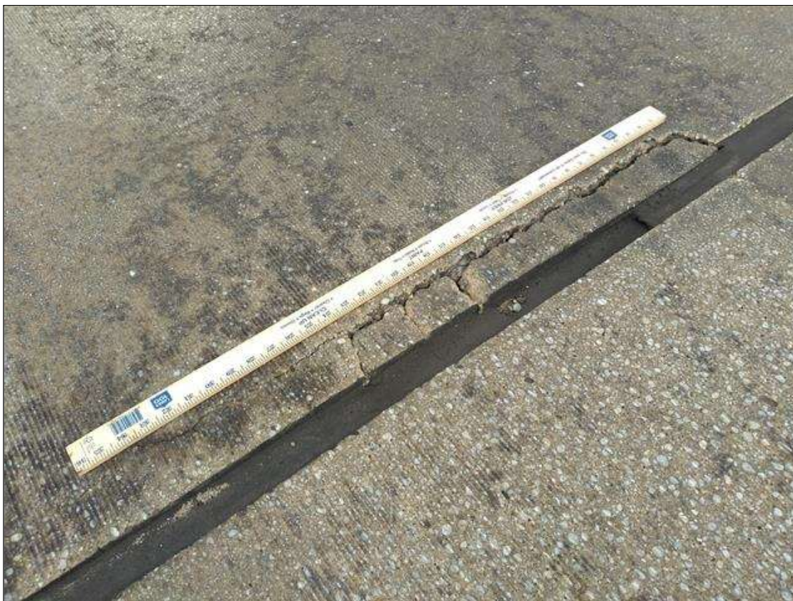
Span 9 Expansion Joint Bent 8: (PAR) AT BENT 8, RIGHT LANE SPALL 4 FOOT WIDE X 2.5 INCH LONG
