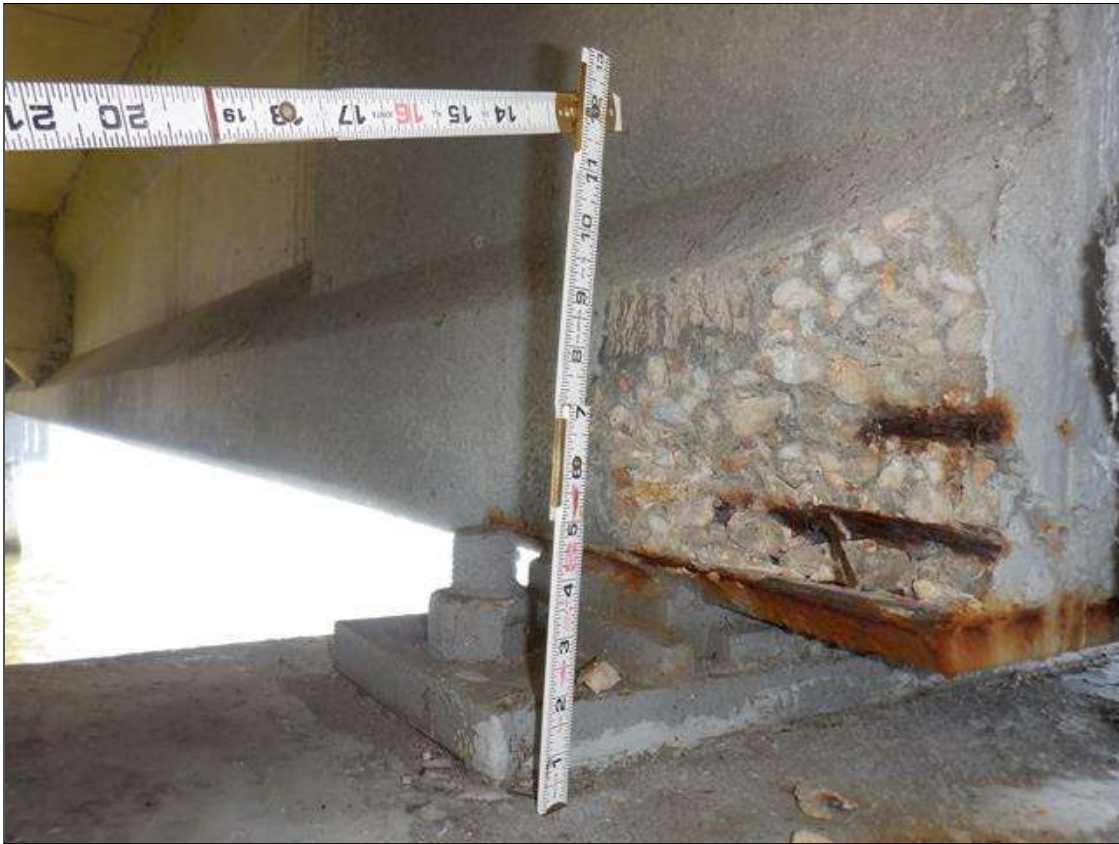
Span 11 Beam 4: (PAR) NORTH FACE BOTTOM FLANGE, AT BENT 10, SPALL (12 INCHES X 7 INCHES X 2 INCHES) WITH (2) EXPOSED RUSTED STRANDS, SECTION LOSS (30 PERCENT) ON BOTTOM STRAND
