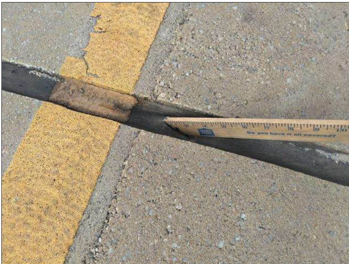
Span 112 Expansion Joint Bent 111: AT BENT 111, AT LEFT SHOULDER, 2 INCH FULL DEPTH TEAR
