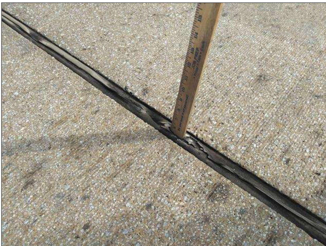
Span 111 Expansion Joint Bent 110: SCATTERED THROUGHOUT BOTH LANES, SEAL DAMAGED AND TORN (28 FEET)
