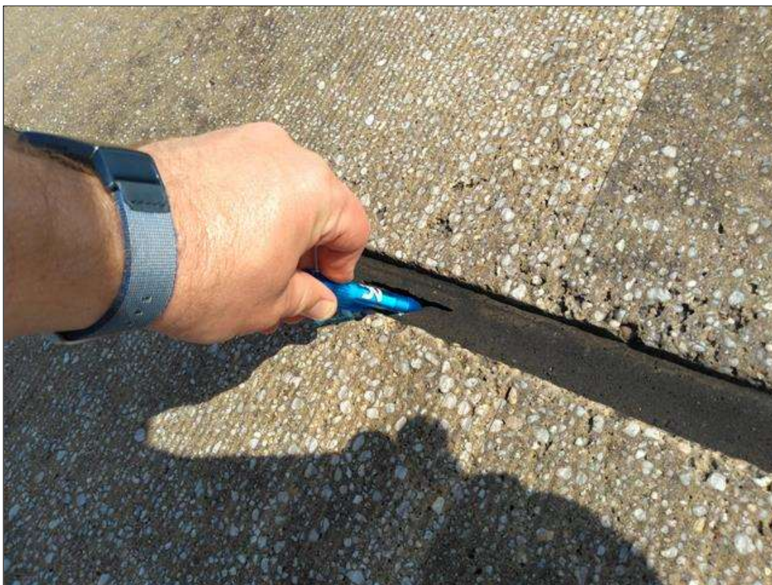
Span 144 Expansion Joint Bent 143: AT BENT 143, LEFT LANE, 2 INCH LONG X FULL DEPTH CRACK
