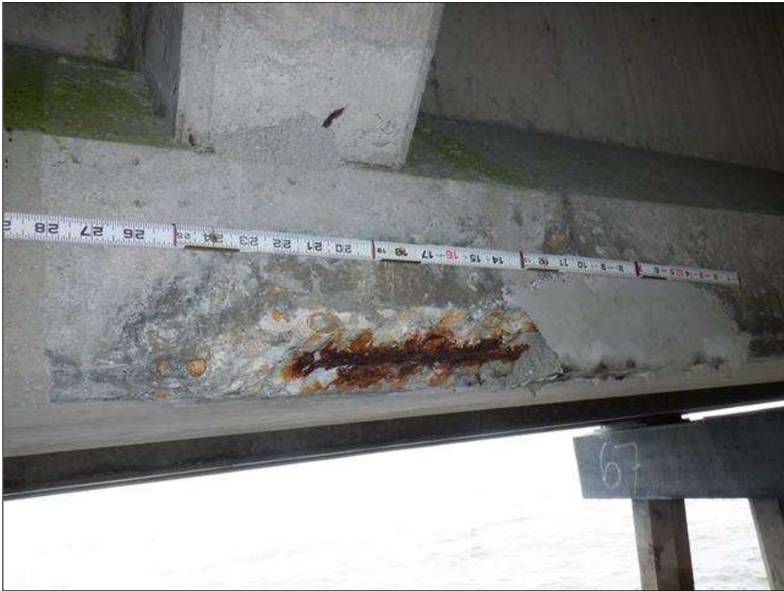
Span 68 Beam 2: (PAR) BOTTOM FLANGE NORTH FACE, 12 FEET FROM BENT 67, FAILED PATCH/SPALL (24 INCHES LONG X 4 INCHES HIGH X 2 INCHES DEEP) WITH EXPOSED RUSTED STRANDS (25 PERCENT SECTION LOSS)
