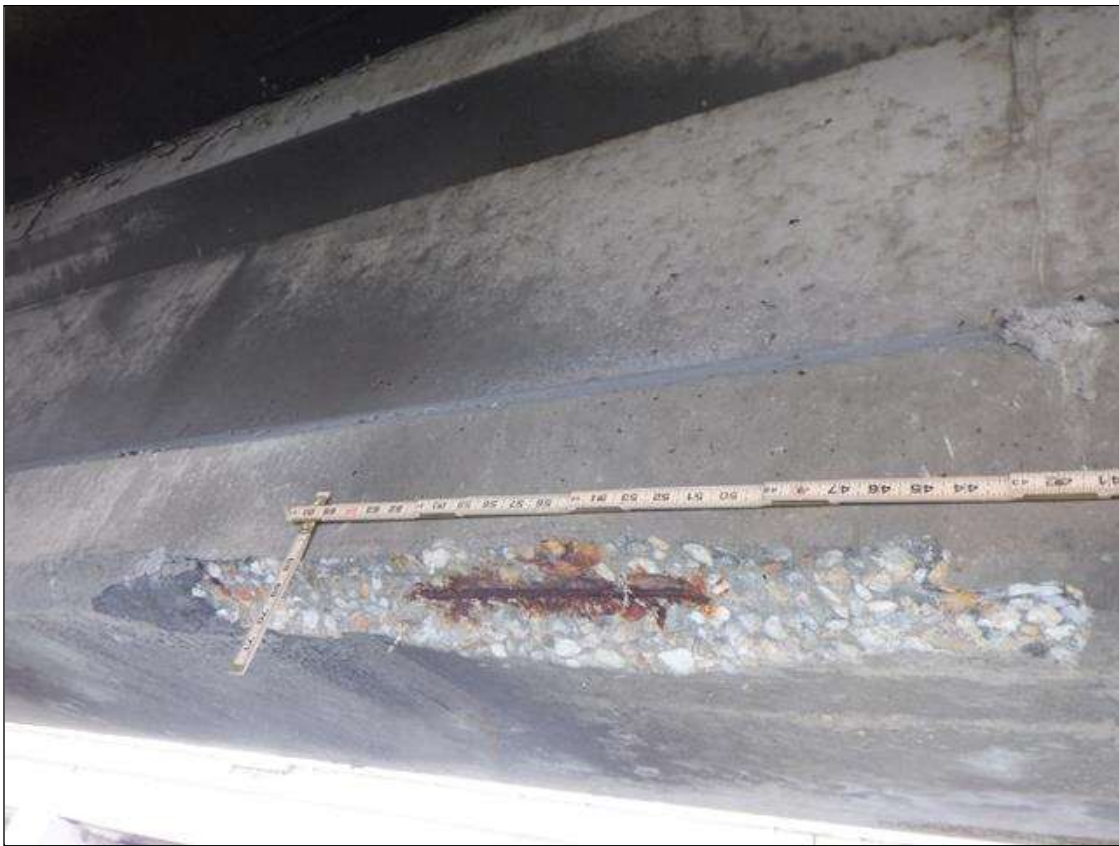
Span 112 Beam 1: (PAR) SOUTH FACE OF BOTTOM FLANGE AT BENT 111, SPALL (36 INCHES LONG X 2 INCHES HIGH X 6 INCHES ON BOTTOM X 1 INCH DEEP) WITH (1) EXPOSED STRAND (10 PERCENT LOSS)
