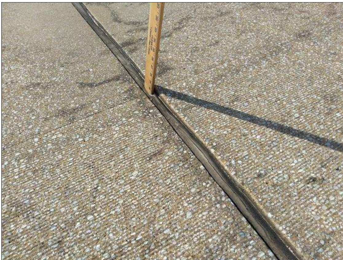
Span 229 Expansion Joint Bent 228: AT BENT 228, FULL WIDTH X FULL DEPTH CRACK
