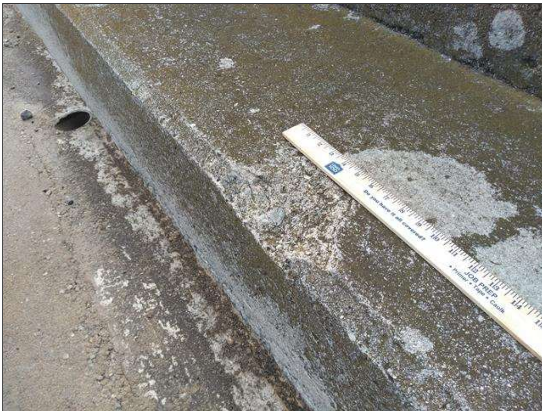
Span 15 Right Bridge Rail: CURB BETWEEN RAILPOSTS 3 AND 4, SPALL (8INCHES X 4INCHES X 2 INCHES)
