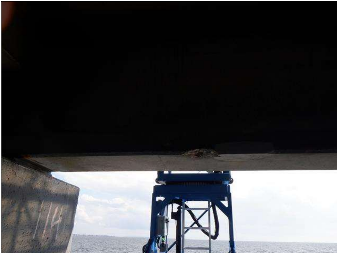
Span 114 Beam 4: UNDERSIDE OF BOTTOM FLANGE 6 FEET FROM BENT 114, SPALL (10 INCHES X 5 INCHES X 1 INCHES) NEXT TO EPOXY PATCHED AREA (18 INCHES X 3 INCHES)
