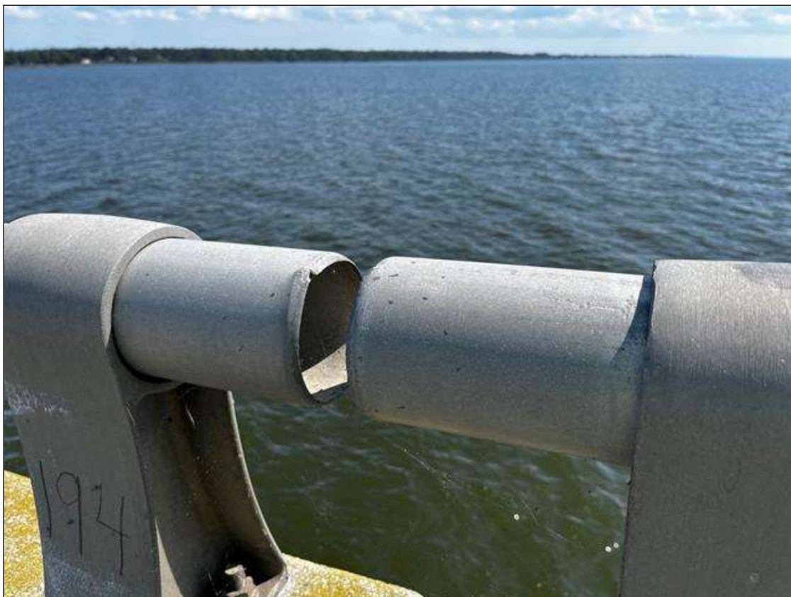
Span 195 Right Bridge Rail: AT RAIL END AT BENT 194, RAILING CAP MISSING
