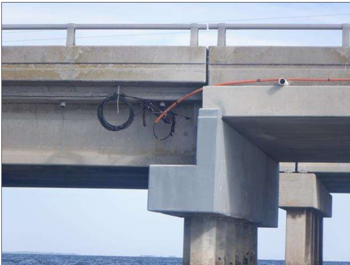
TYPICAL BEAM OVER INTERIOR BENT, BENT 153 IN VIEW
