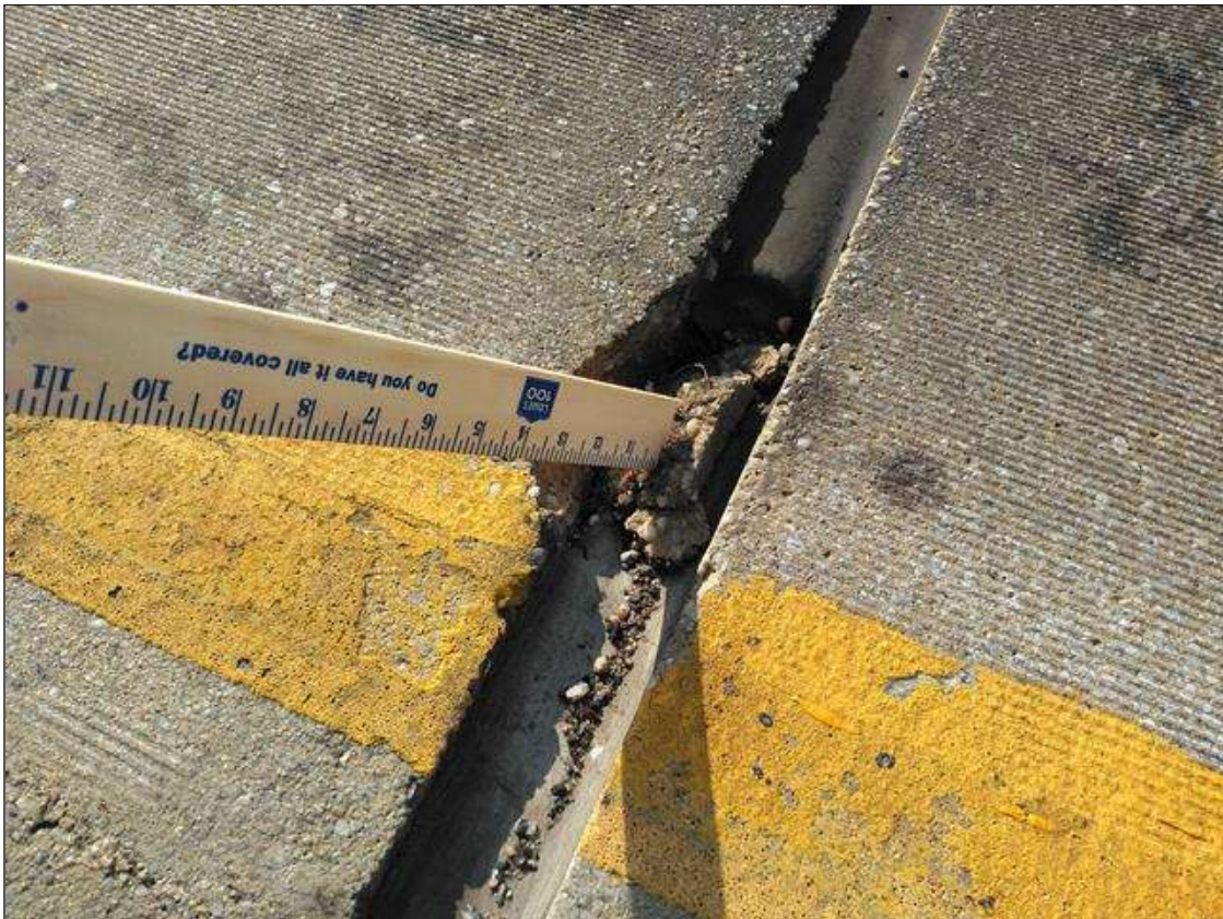
Span 1 Expansion Joint End Bent 1: AT END BENT 1 JOINT, LEFT EDGE OF TRAVEL, EDGE SPALL 6 INCH LONG X 1 INCH WIDE. NO SEAL OF JOINT MATERIAL.
