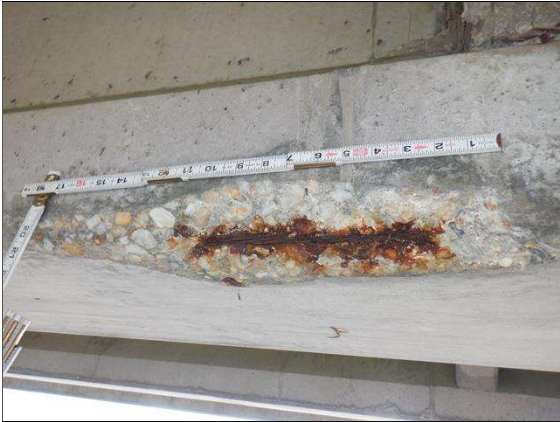
Span 69 Beam 2: (PAR) NORTH FACE OF BOTTOM FLANGE, AT 20 FEET FROM BENT 68, SPALL (16 INCHES X 3 INCHES X 2 INCHES) WITH EXPOSED STRANDS (30 PERCENT SECTION LOSS) ON STRAND
