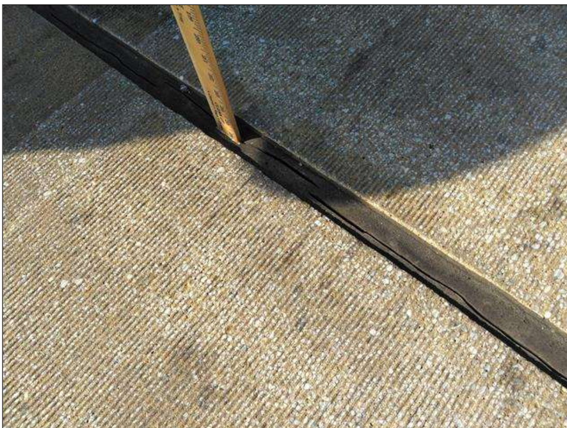
Span 218 Expansion Joint Bent 217: AT BENT 217, CRACK FULL DEPTH
