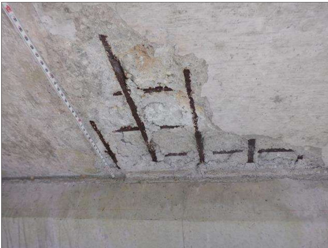
Span 192 Deck: (PAR) UNDERSIDE OF DECK IN BAY 3 AT 24 FEET FROM BENT 192, SPALL (3 FEET X 2 FEET X UP TO 2 INCHES DEEP) WITH EXPOSED RUSTED REINFORCING (10 PERCENT LOSS) SECOND MAT EXPOSED
