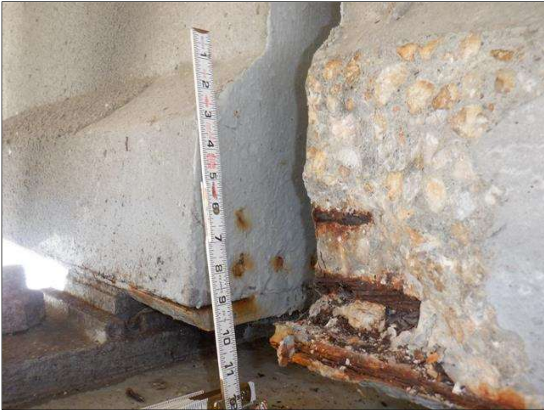
Span 77 Beam 3: (PAR) NORTH FACE OF BOTTOM FLANGE, AT BENT 77, SPALL (6 INCHES X 8 INCHES X 2 INCHES) WITH EXPOSED STRANDS (10 PERCENT SECTION LOSS)
