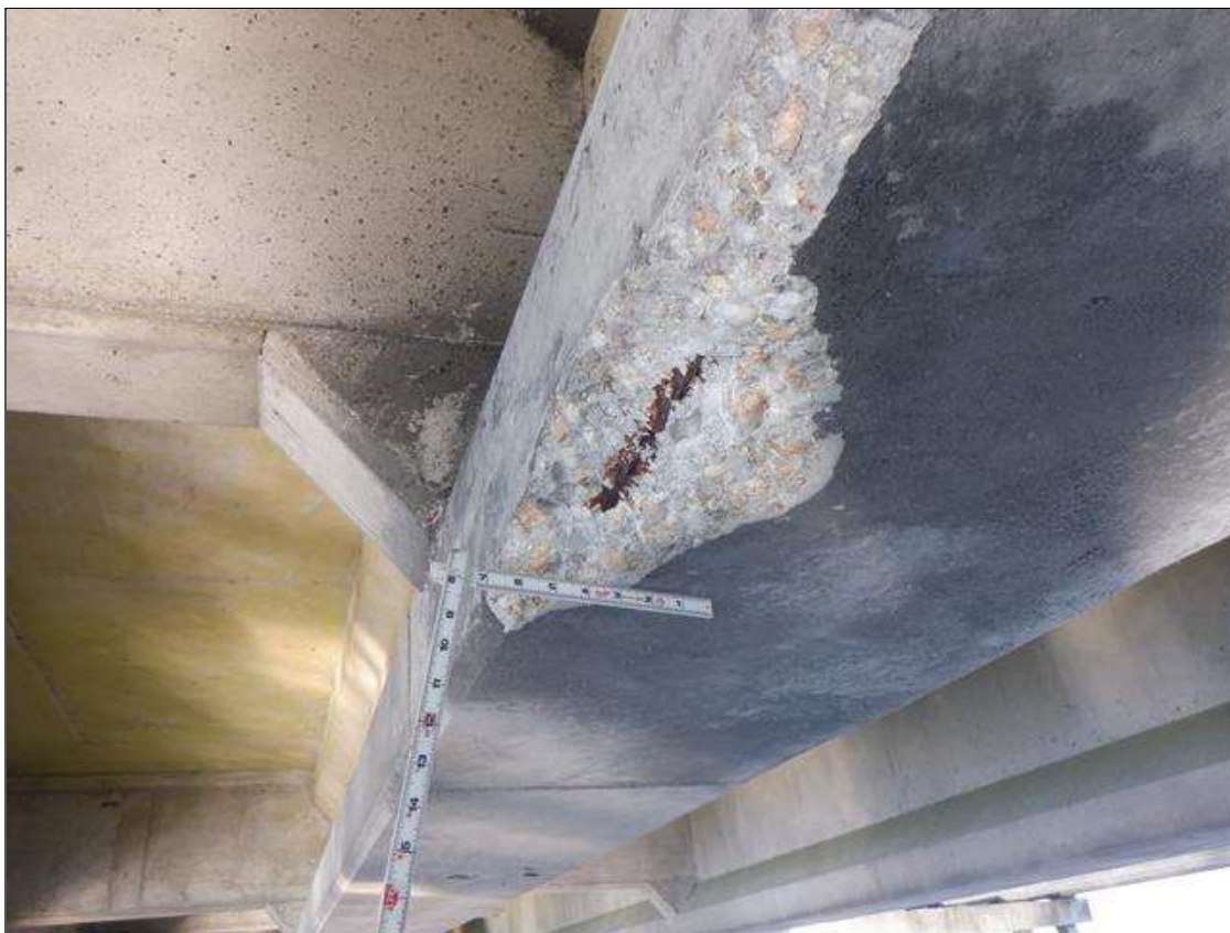
Span 238 Beam 2: (PAR) BOTH FACES OF BOTTOM FLANGE AT 20 FEET FROM BENT 238, PATCHED AREA (2 FEET LONG X 6 INCHES WIDE X 2 INCHES DEEP) WITH ONE (1) EXPOSED RUSTED STRAND (10 PERCENT SECTION LOSS)
