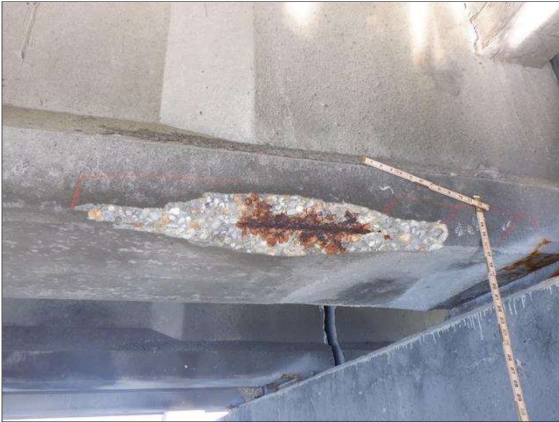
Span 109 Beam 3: (PAR) SOUTH FACE OF BOTTOM FLANGE 4 FEET FROM BENT 109, DELAMINATION/SPALL (40 INCHES LONG X 5 INCHES HIGH X 2 INCHES DEEP WITH (1) EXPOSED AND SEVERED STRAND
