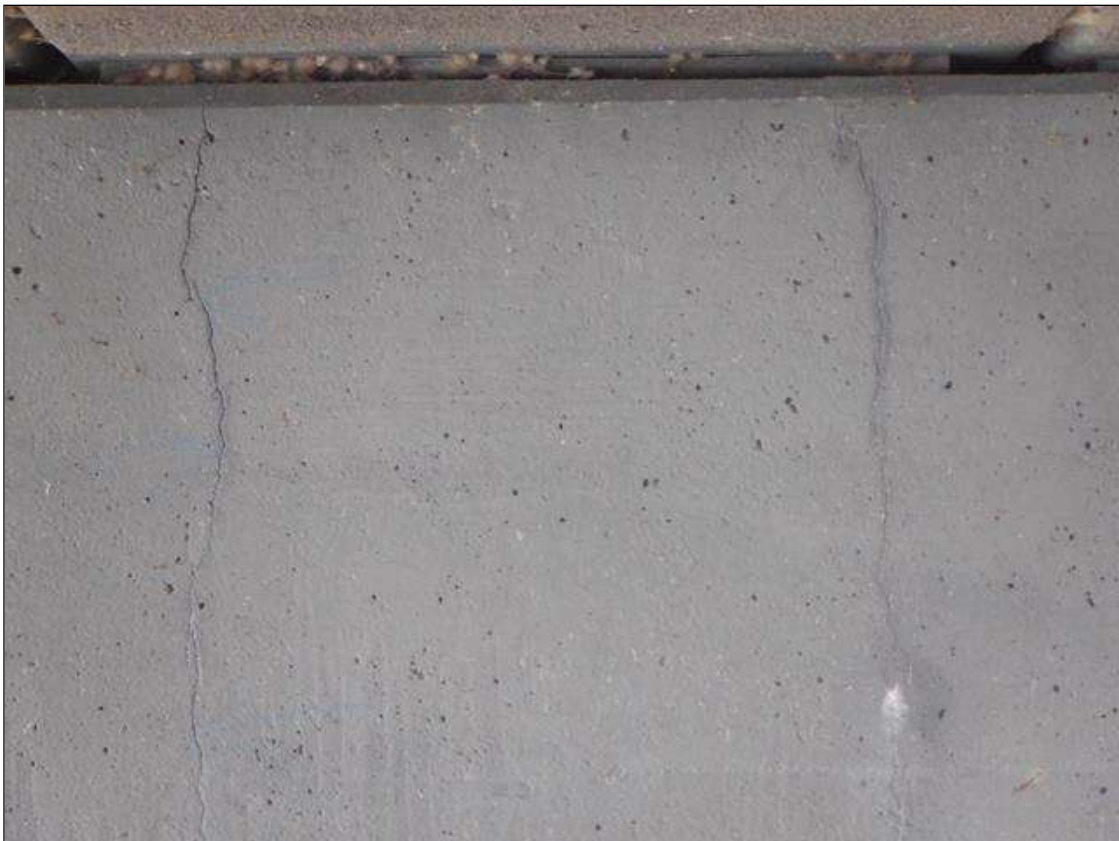
Bent 153 Cap 1: TOP OF EAST FACE SCATTERED THROUGHOUT, (5) VERTICAL CRACKS (UP TO 3 FEET X 1/16 INCHES) SOME WITH EFFLORESCENCE
