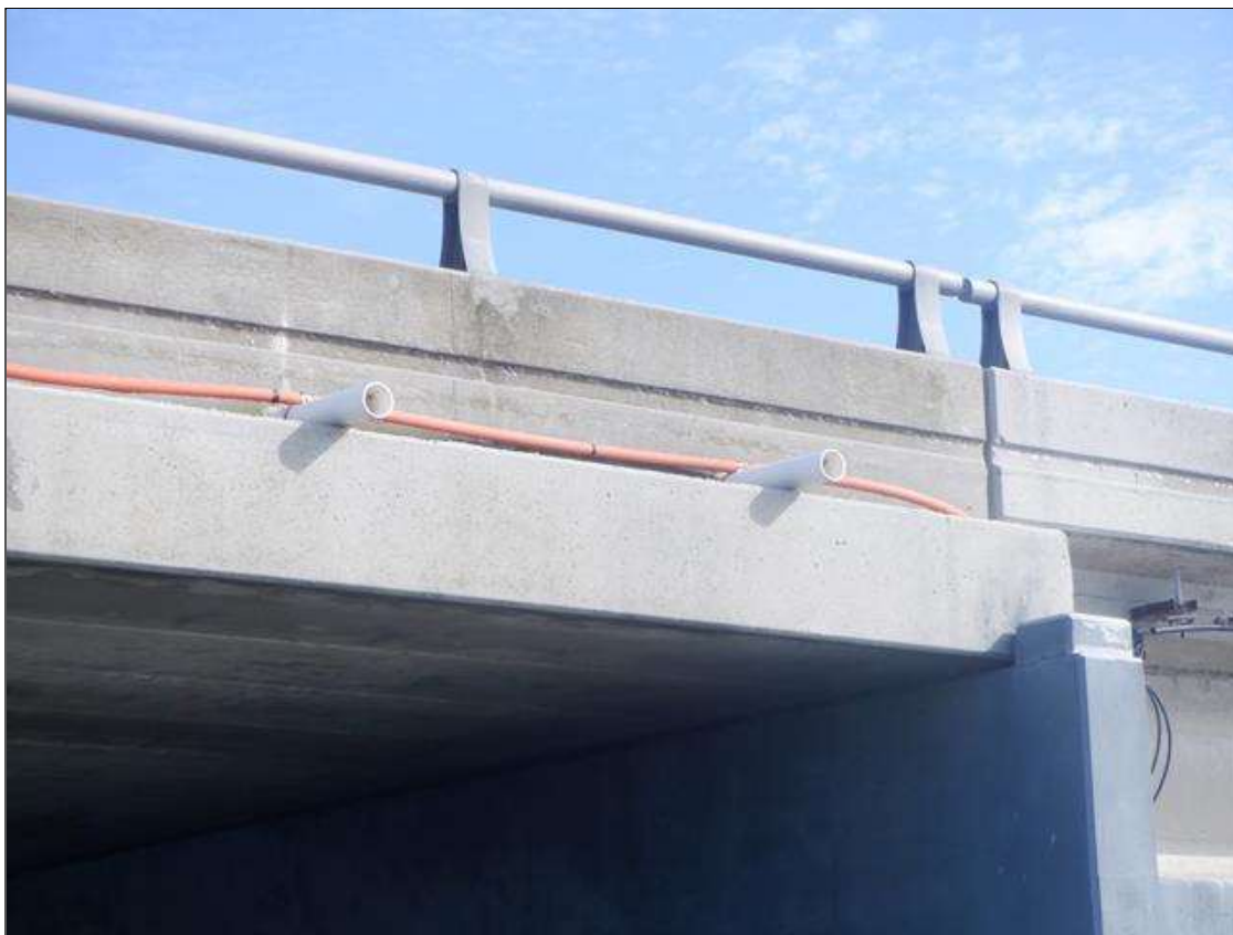
ATTACHED UTILITY, SPAN 154 IN VIEW
