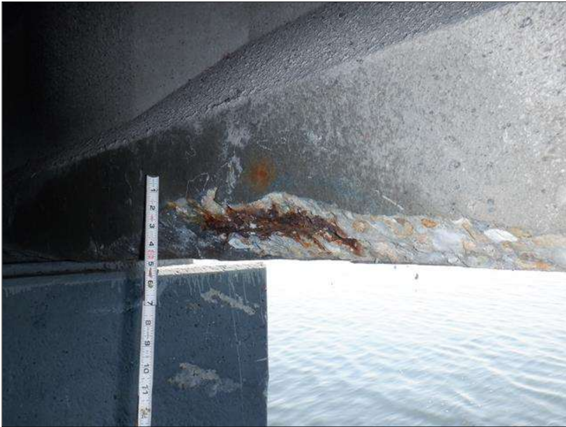
Span 157 Beam 4: (PAR) NORTH FACE OF BOTTOM FLANGE AT 4 FEET FROM BENT 157, FAILED PATCH/SPALL (36 INCHES X 4 INCHES HIGH X UP TO 2 INCHES DEEP) WITH EXPOSED RUSTED STRANDS (10 PERCENT SECTION LOSS)
