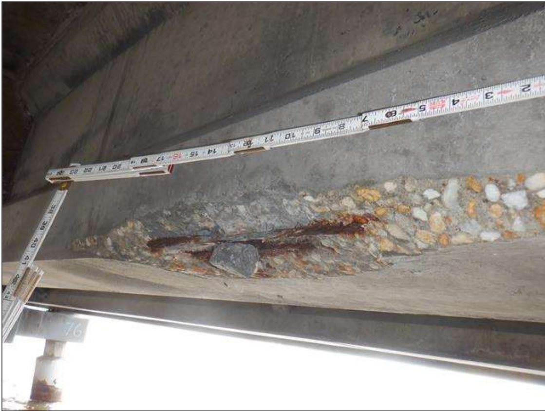
Span 76 Beam 2: (PAR) NORTH FACE OF BOTTOM FLANGE, AT 12 FEET FROM BENT 75, FAILED PATCH/SPALL (36 INCHES X 3 INCHES X 1 INCHES) WITH EXPOSED STRANDS (50 PERCENT SECTION LOSS)
