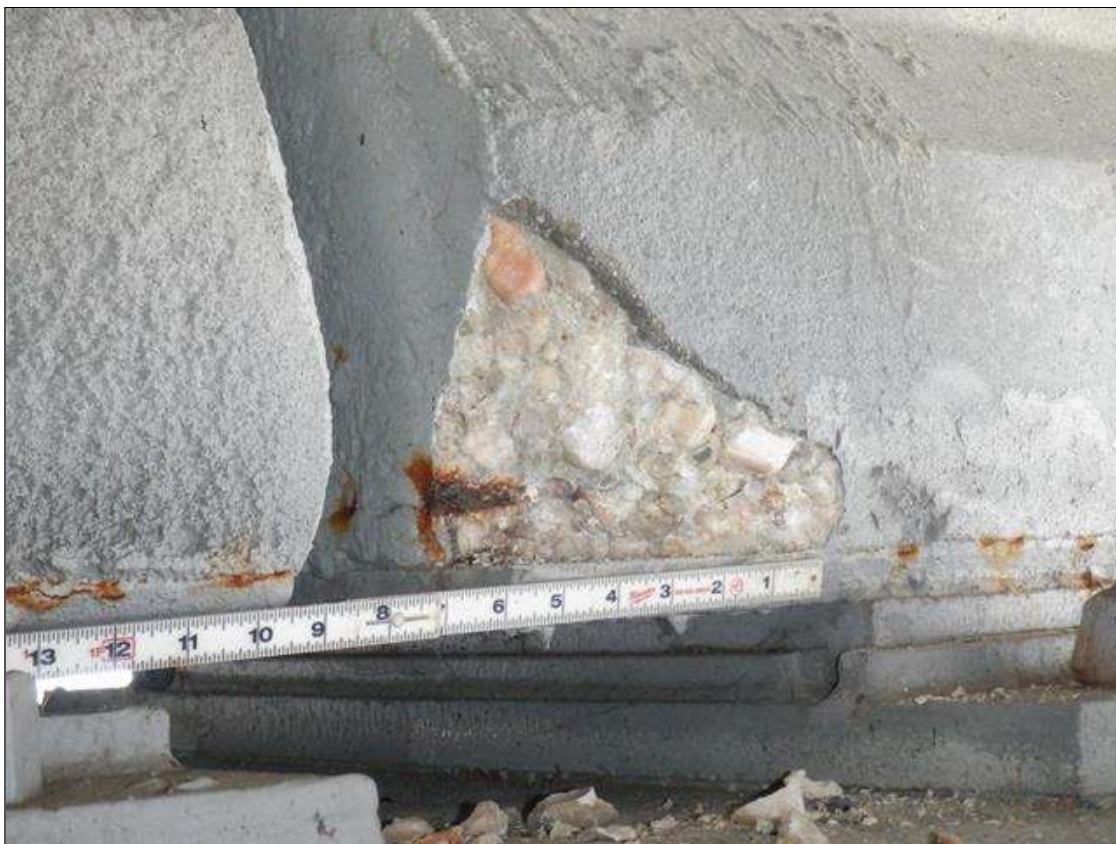
Span 9 Beam 2: SOUTH FACE BOTTOM FLANGE AT BENT 8, SPALL (6 INCHES X 4 INCHES X UP TO 2 INCHES DEEP) WITH EXPOSED RUSTED STRAND (NO SECTION LOSS)
