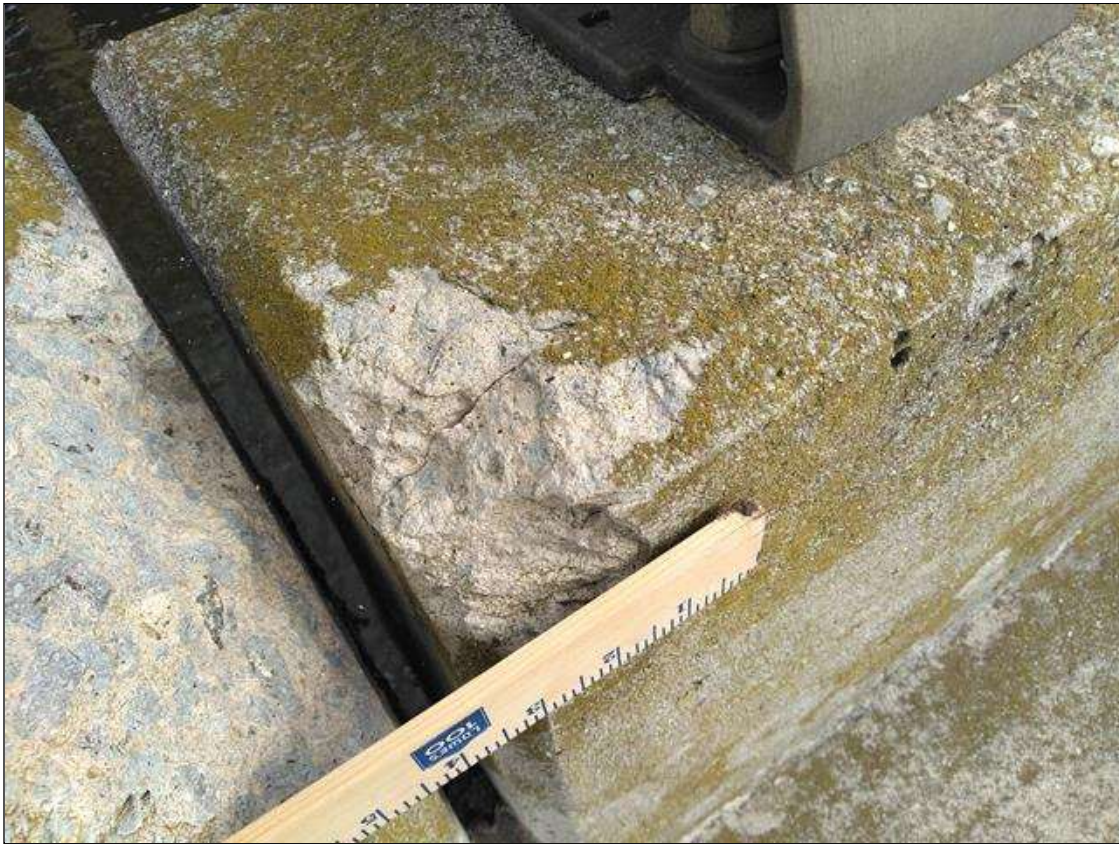
Span 6 Left Bridge Rail: AT BENT 5, SPALL (6INCHES X 6INCHES X 1/2 INCHES)
