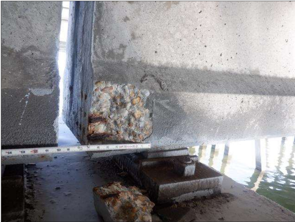
Span 169 Beam 1: (PAR) SOUTH FACE OF BOTTOM FLANGE BENT 168, SPALL (7 INCHES X 7 INCHES X 2.5 INCHES) WITH 2 (TWO) EXPOSED STRANDS (5 PERCENT SECTION LOSS) ON STRAND
