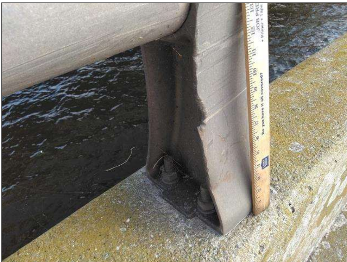
Span 116 Left Bridge Rail: IMPACT DAMAGE TO POST 4
