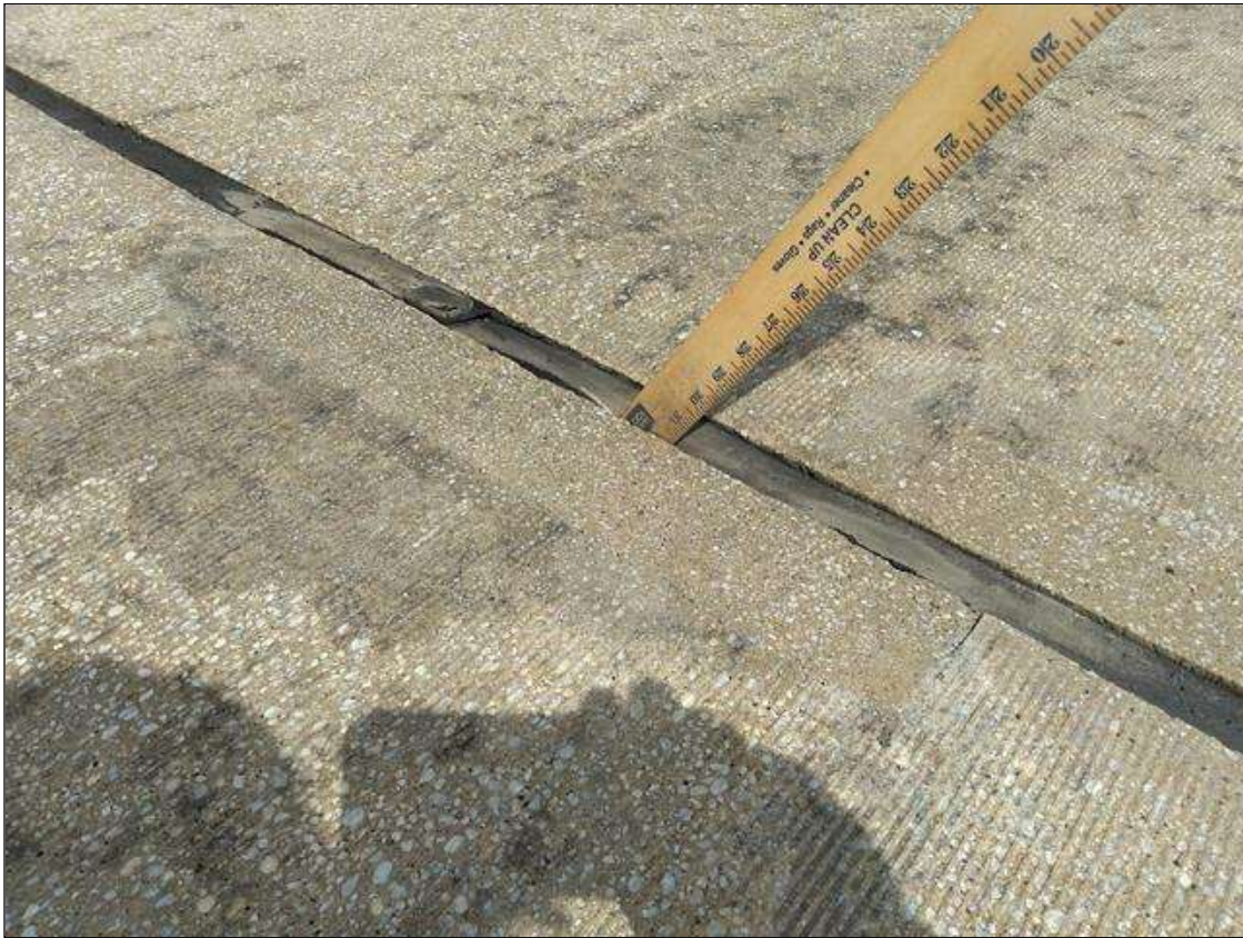
Span 68 Expansion Joint Bent 67: LEFT LANE NEAR CENTERLINE OF ROADWAY, (2) PATCHED AREAS (UP TO 1FEET X 6 INCHES). NO ADHESION AT PATCHES
