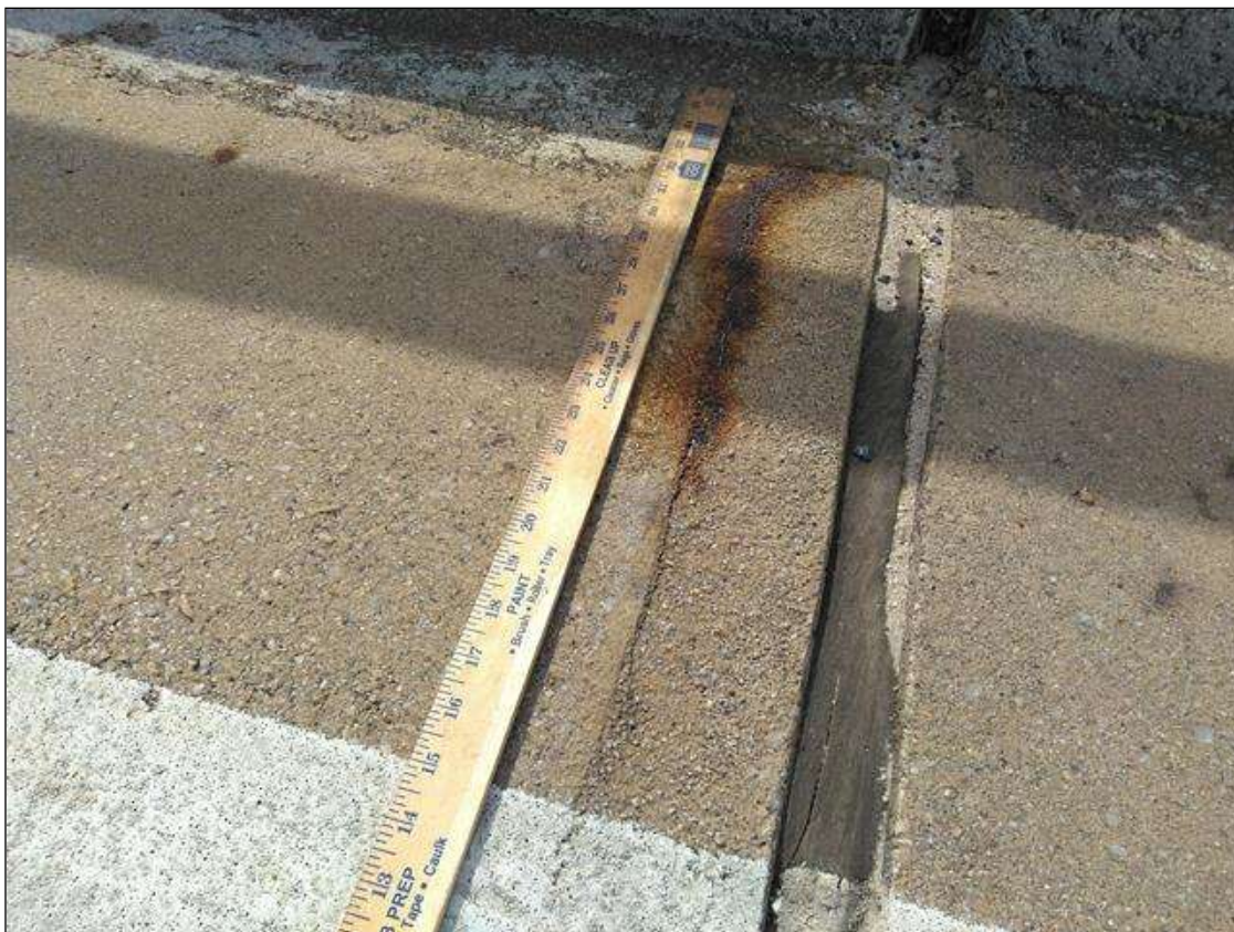
Span 221 Expansion Joint Bent 220: AT BENT 220, RIGHT SHOULDER, UNSOUND PATCH 2 FOOT X 4 INCH WITH RUST STAINING
