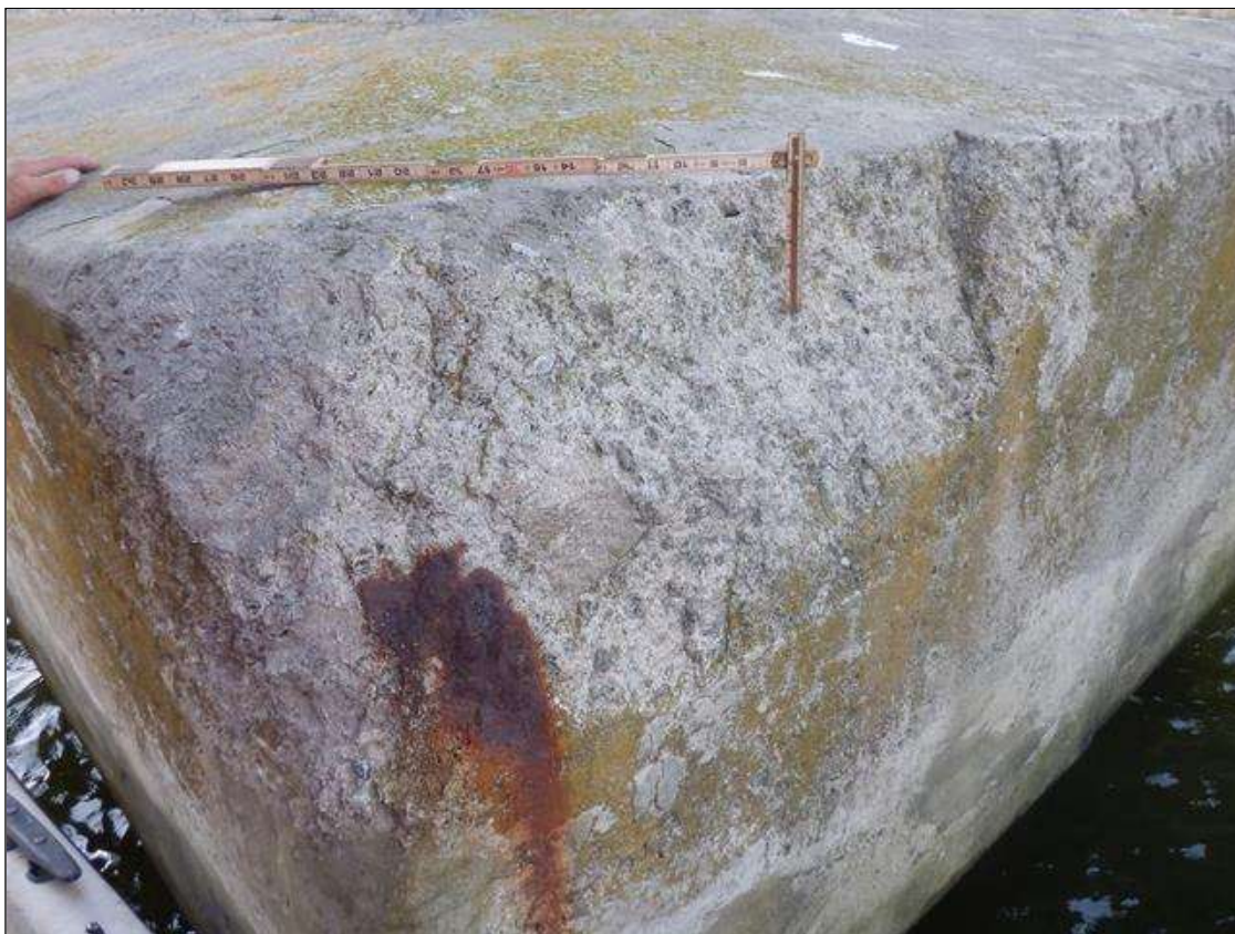
Bent 181 Footing: NORTHEAST CORNER, SPALL (5FEET X 18INCHES X 3 INCHES) WITH EXPOSED RUSTED REBAR
