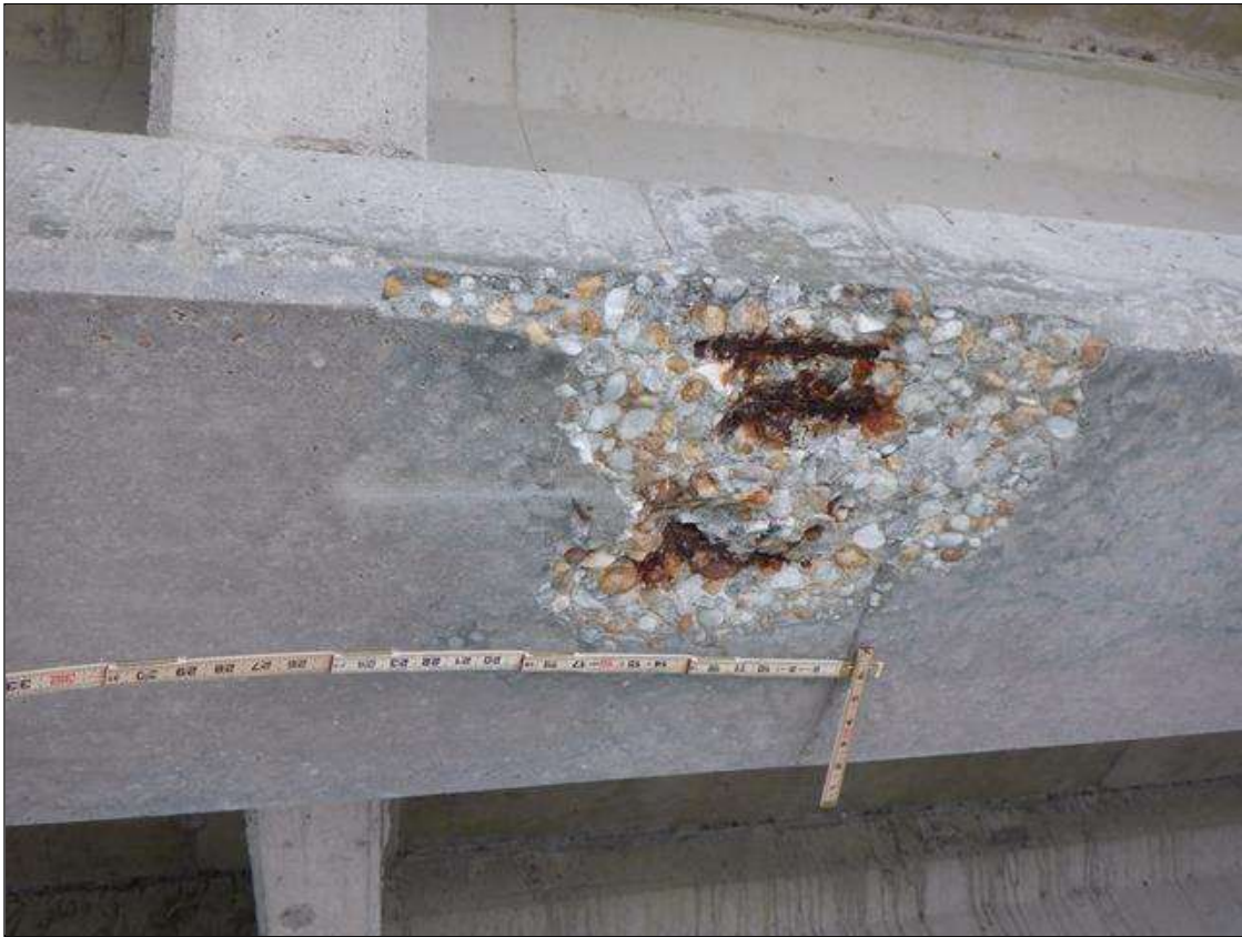
Span 143 Beam 2: (PAR) BOTTOM OF BOTTOM FLANGE AT MIDSPAN, (22 INCHES LONG X 13 INCHES WIDE X 1.5 INCHES DEEP) WITH (3) THREE EXPOSED STRANDS (10 PERCENT LOSS)
