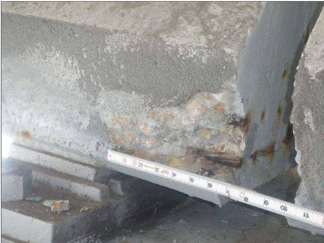
Span 169 Beam 2: (PAR) NORTH FACE OF BOTTOM FLANGE AT BENT 168, SPALL (6 INCHES X 5 INCHES UP TO 2 INCHES DEEP) WITH TWO (2) EXPOSED STRANDS (NO SECTION LOSS)
