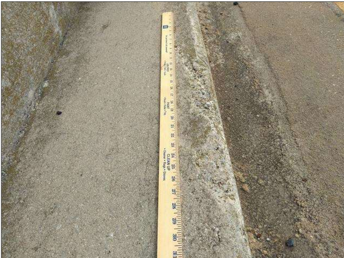
Span 13 Left Bridge Rail: TOP CORNER OF CURB AT BENT 12, SPALL (3FEET X 1INCHES X 1 INCHES)
