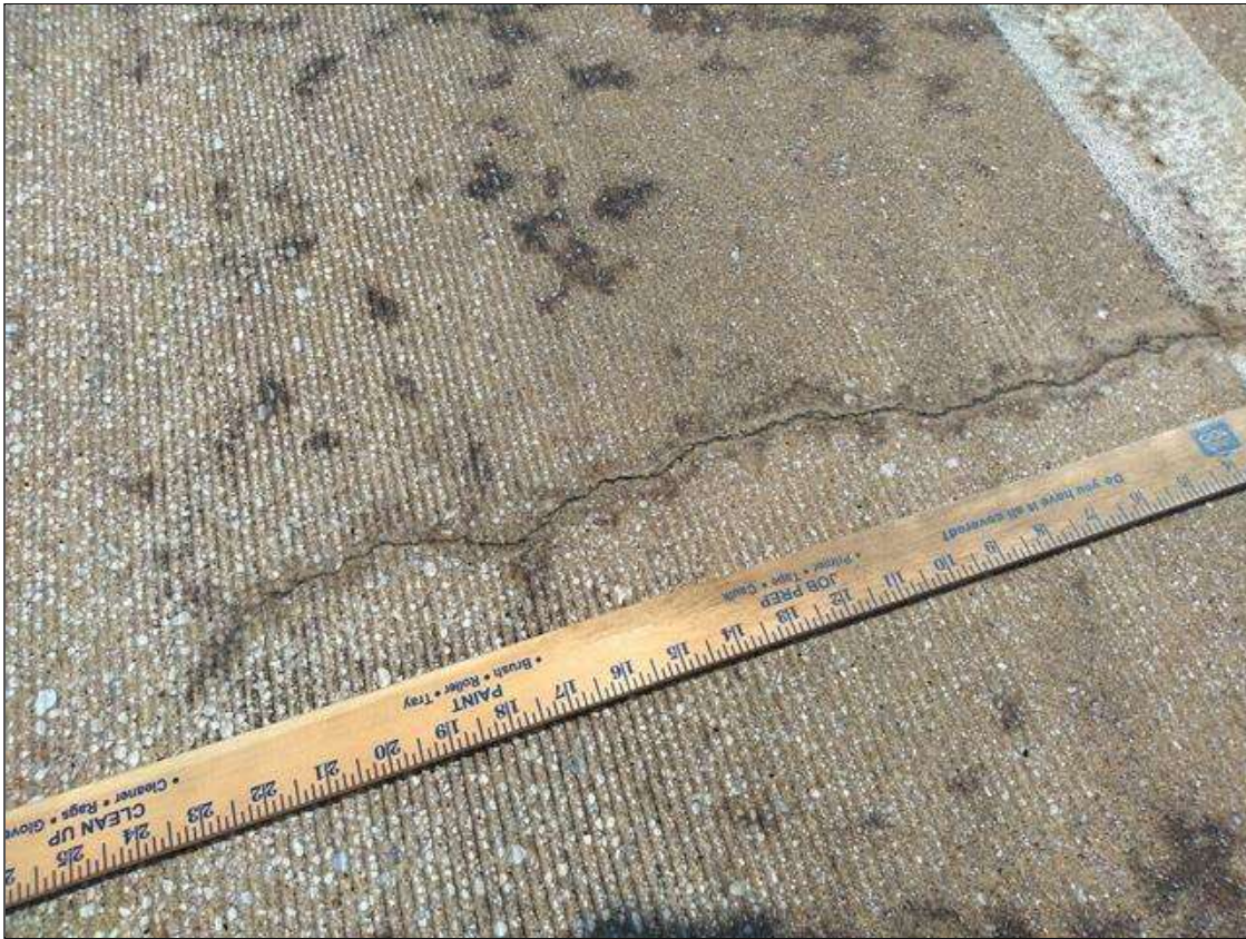
Span 139 Deck: WITHIN 8 FEET OF BENT 139 IN RIGHT SHOULDER (2) 2 FOOT X 0.06 INCH TRANSVERSE CRACKS
