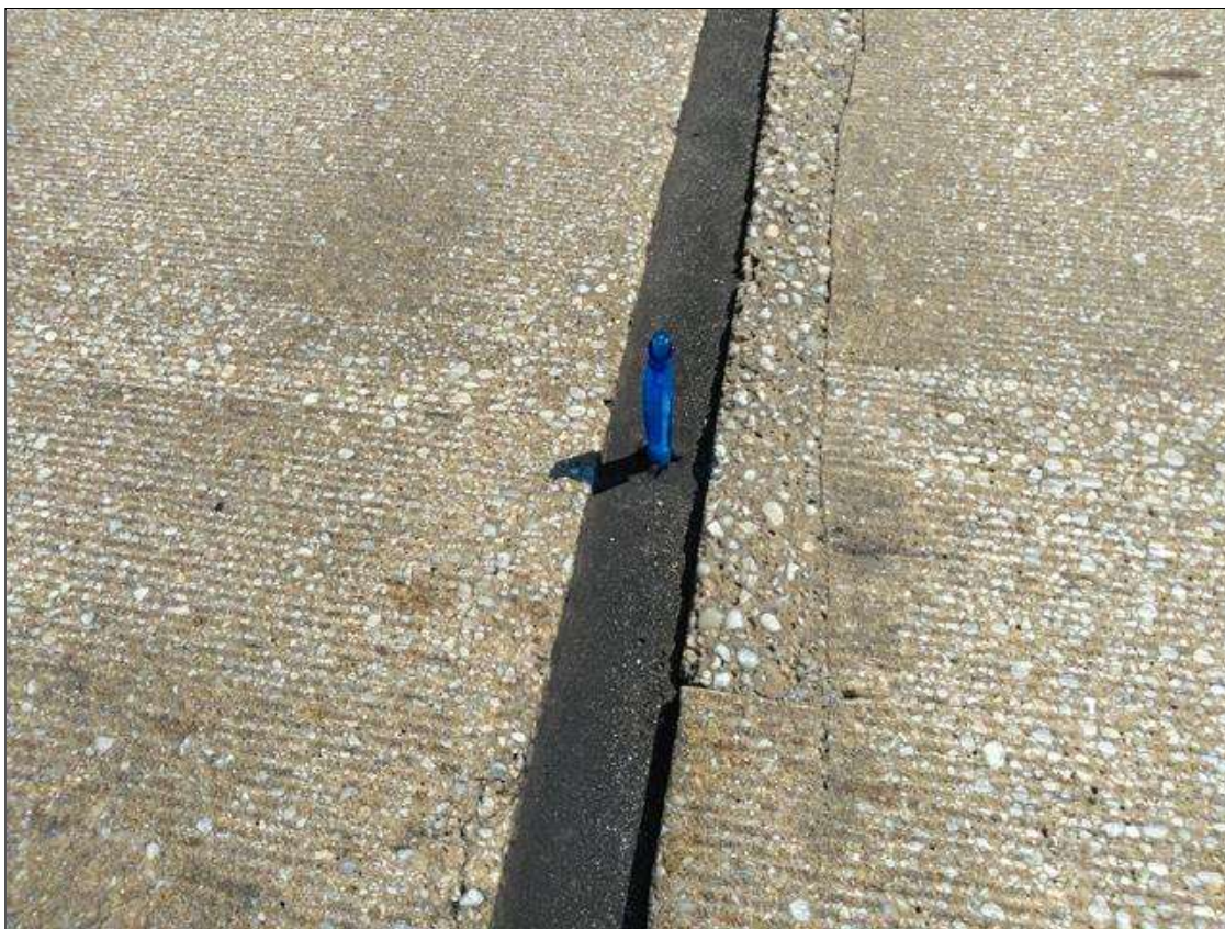
Span 194 Expansion Joint Bent 193: AT BENT 193, CENTER OF RIGHT LANE CRACK PARTIAL DEPTH 2 INCHES WIDE
