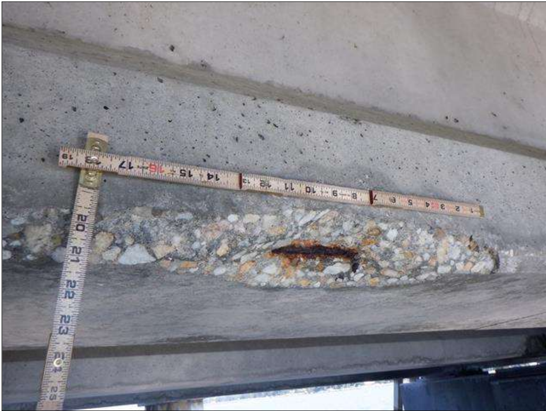
Span 222 Beam 3: (PAR) SOUTH FACE OF BOTTOM FLANGE, AT 18 FEET BENT 222, SPALL (18 INCHES X 5 INCHES X 2 INCHES) WITH EXPOSED RUSTED STRAND (10 PERCENT SECTION LOSS)
