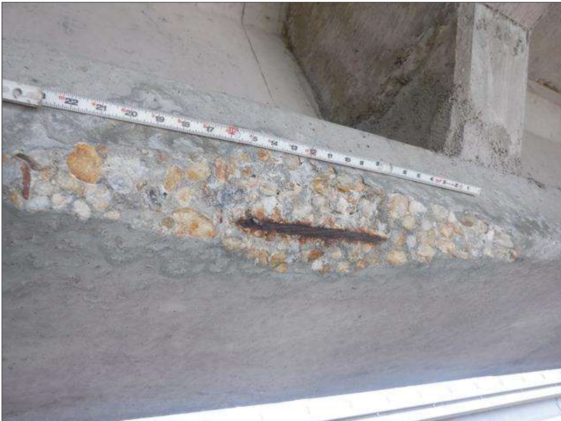
Span 190 Beam 1: (PAR) NORTH FACE OF BOTTOM FLANGE AT MIDSPAN, SPALL (2 FEET X 4 INCHES X 2 INCHES DEEP) WITH ONE (1) EXPOSED STRAND (10 PERCENT LOSS)
