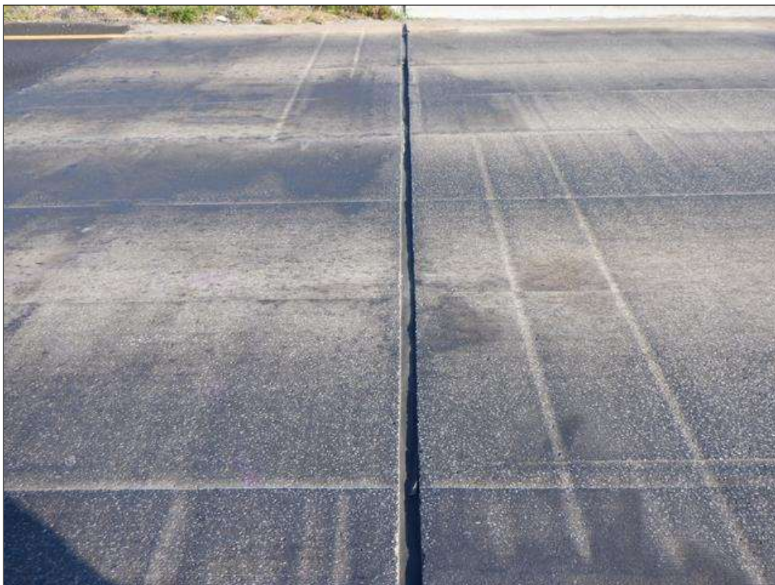
TYPICAL JOINT OVER END BENT, JOINT OVER END BENT 1 IN VIEW
