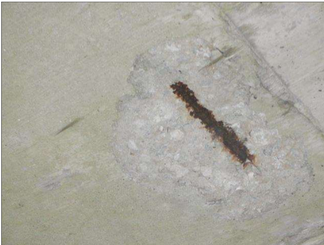
Span 167 Deck: 15 FEET FROM BENT 167 IN BAY 2, SPALL (1 FOOT DIAMETER X 1/2 INCH DEEP)
