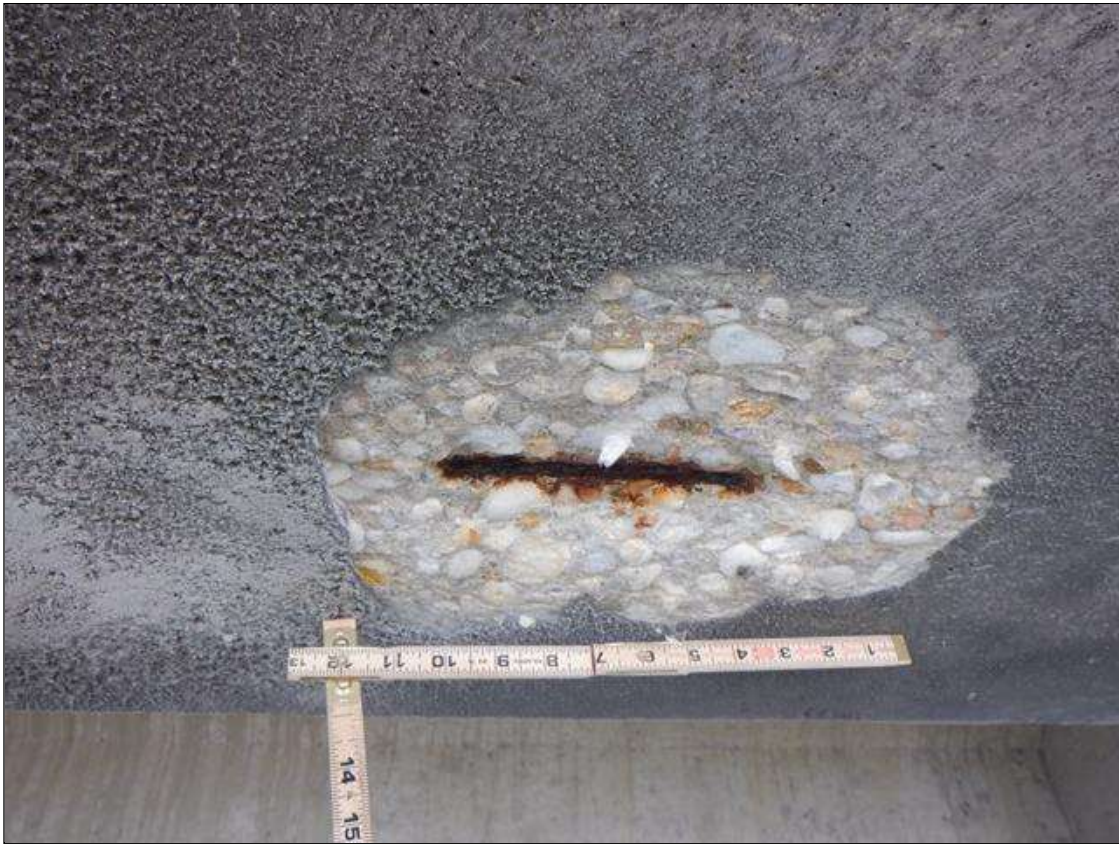
Span 228 Beam 2: (PAR) BOTTOM OF BOTTOM FLANGE AT 24 FEET FROM BENT 228, FAILED PATCH/SPALL (12 INCH DIAMETER X 1 INCH DEEP) WITH EXPOSED RUSTED STRAND (10 PERCENT SECTION LOSS)
