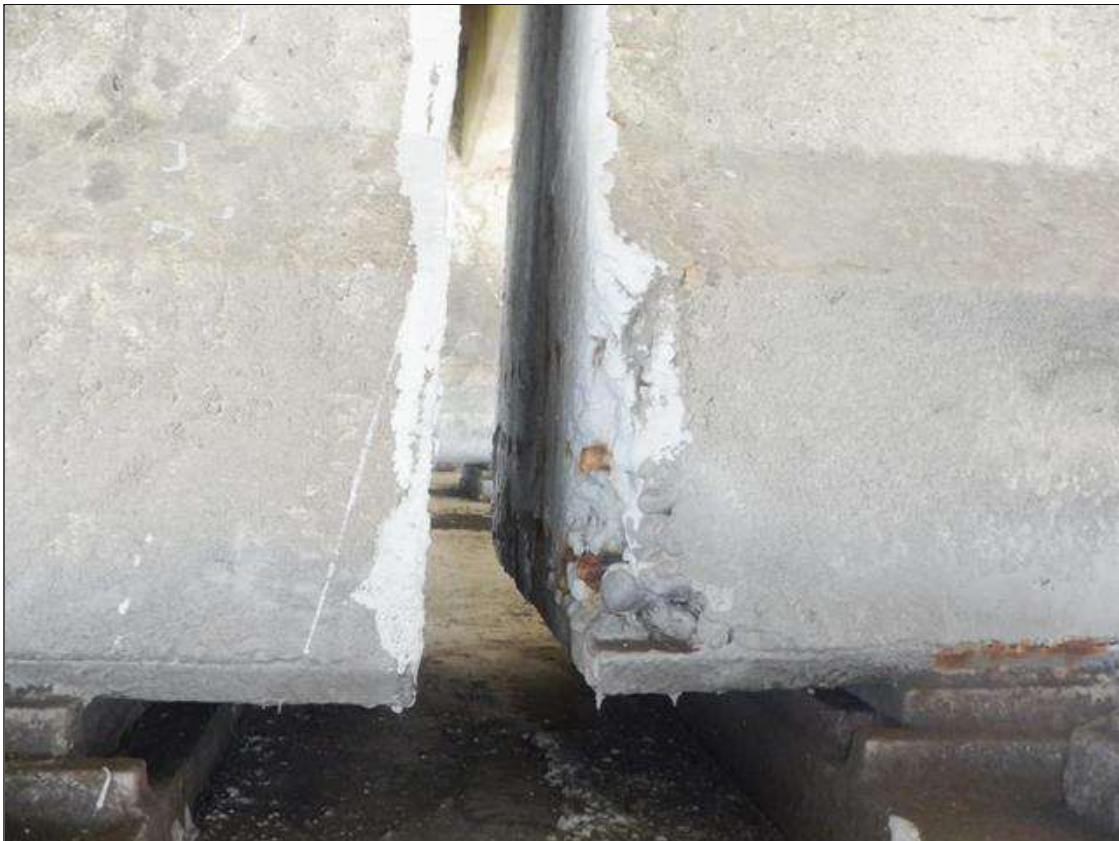
Span 171 Beam 3: (PAR) SOUTH FACE OF BOTTOM FLANGE AT BENT 170, SPALL (3 INCHES X 7 INCHES X 1 INCHES) WITH EXPOSED STRANDS (10 PERCENT SECTION LOSS) ON STRAND
