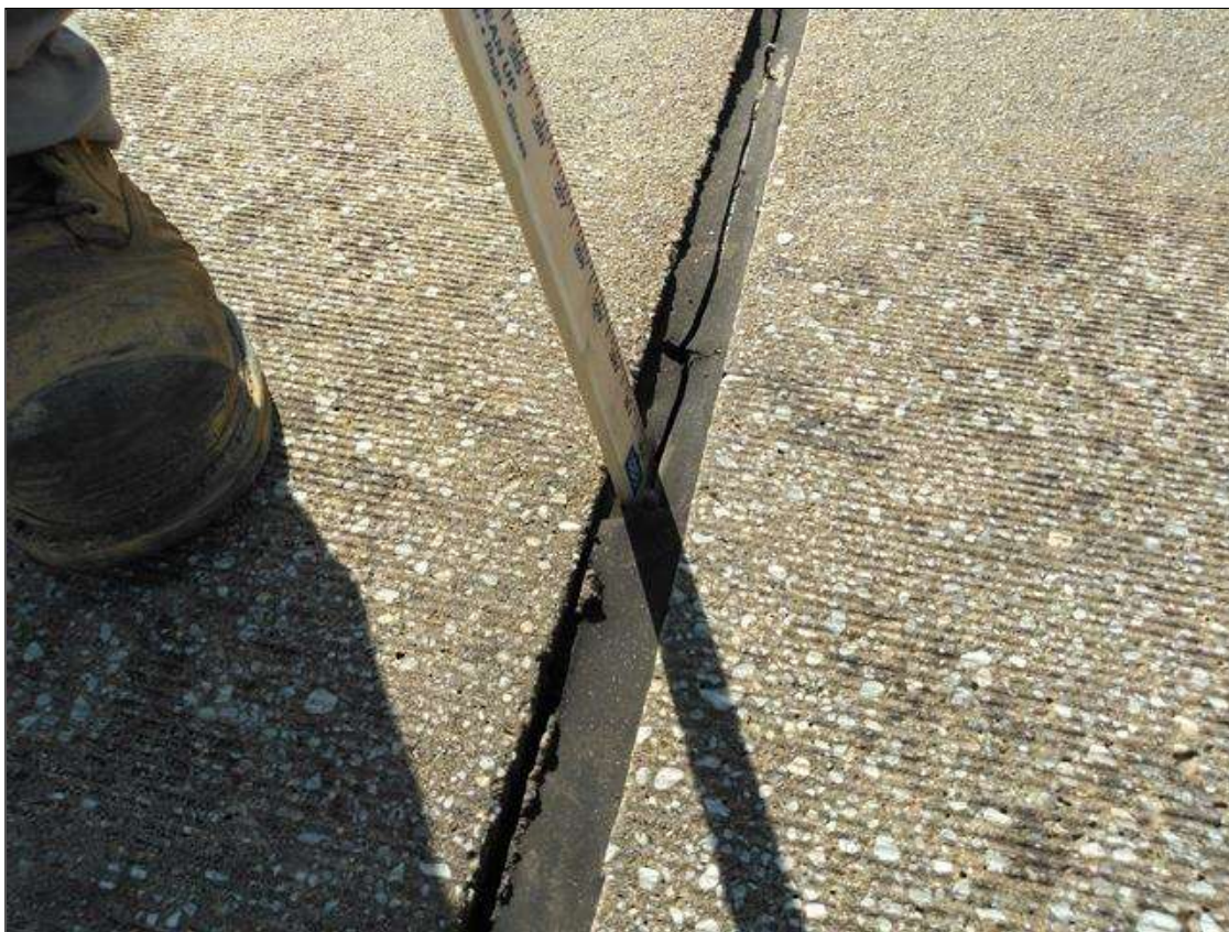
Span 24 Expansion Joint Bent 23: INTERMITTENT THROUGHOUT, SEAL DAMAGE
