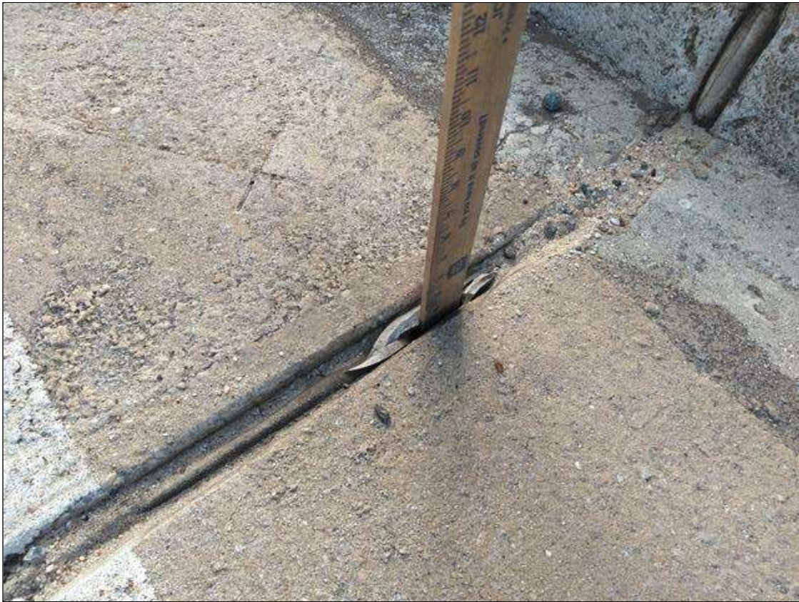
Span 208 Expansion Joint Bent 207: AT BENT 207, PARTIAL DEPTH CRACKING IN SHOULDERS AND CENTERLINE
