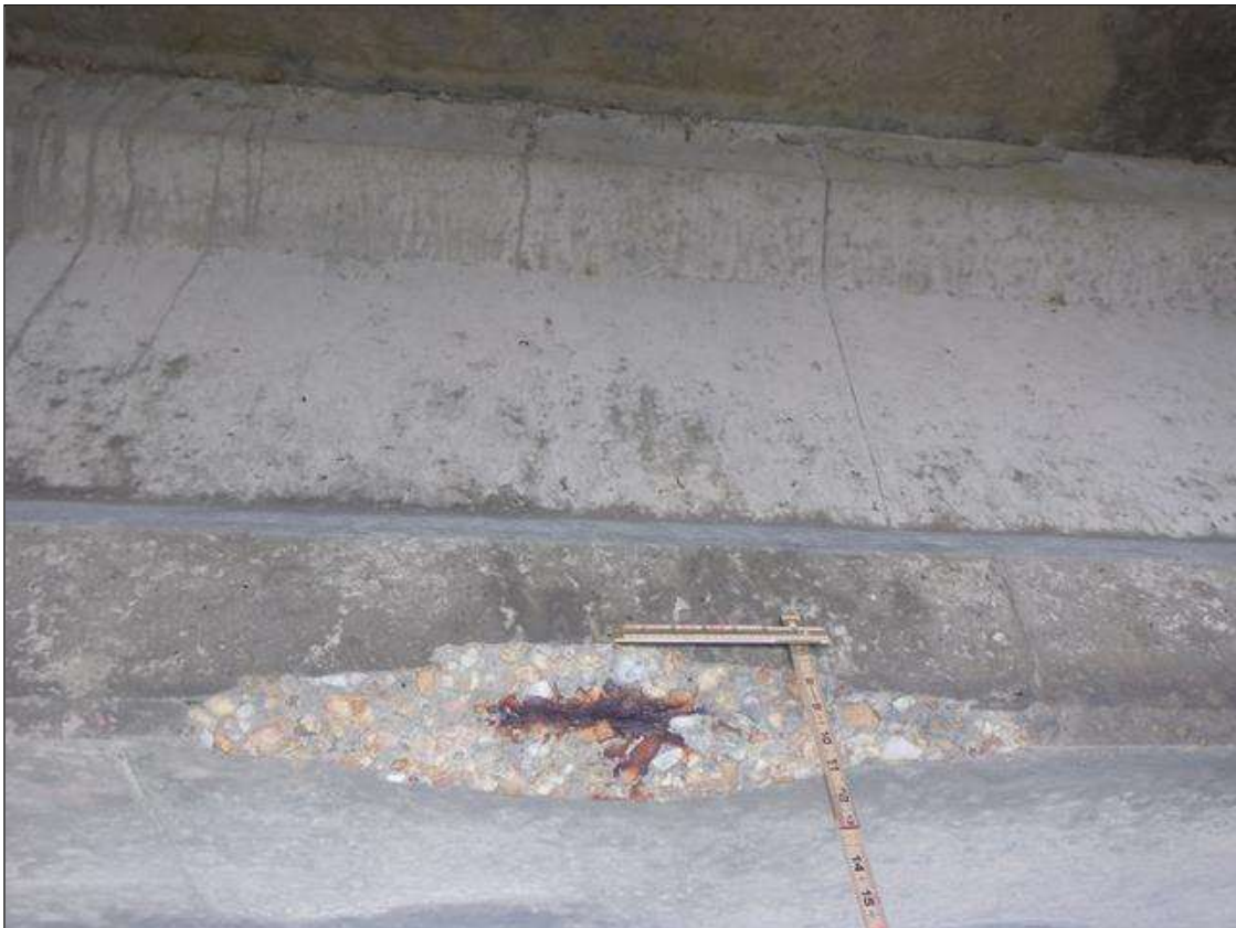
Span 136 Beam 1: (PAR) SOUTH FACE OF BOTTOM FLANGE AT 12FEET FROM BENT 135, SPALL (25INCHES X 5INCHES X 2 INCHES) WITH EXPOSED STRANDS (10 PERCENT SECTION LOSS) ON STRAND
