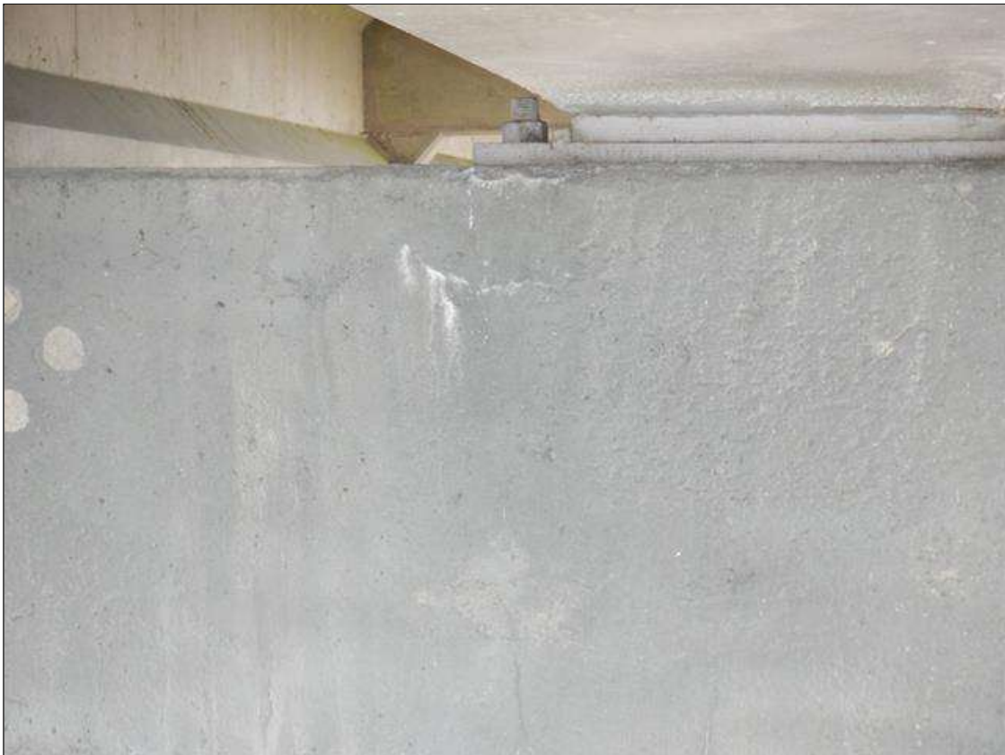
Bent 14 Cap 1: ALL FACES, SCATTERED PATCHED AREAS WITH MAP CRACKING (UP TO 1/32 INCHES), SOME WITH EFFLORESCENCE
