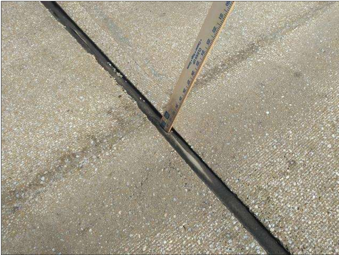
Span 30 Expansion Joint Bent 29: AT BENT 29, INTERMITTENT FULL DEPTH CRACKS IN JOINT
