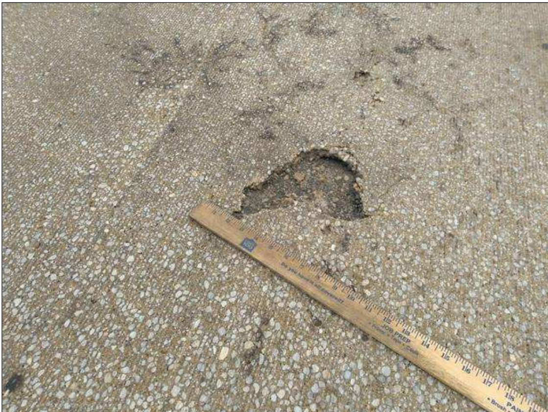
Span 86 Deck: RIGHT LANE AT 16 FEET FROM BENT 86, SPALLS (8 INCHES X 6 INCHES X 1/2 INCHES) AND 3 INCH X 1 INCH X 0.50 INCH DEEP
