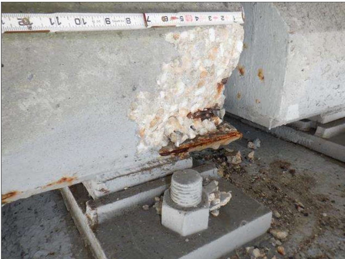
Span 16 Beam 3: (PAR) SOUTH FACE BOTTOM FLANGE, AT BENT 16, SPALL (8 INCHES X 7 INCHES X 2 INCHES) WITH (2) EXPOSED RUSTED STRANDS, SECTION LOSS (20 PERCENT) ON BOTTOM STRAND
