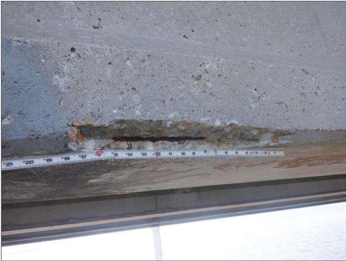
Span 171 Beam 1: BOTH FACES OF BOTTOM FLANGE AT 15 FEET FROM BENT 171, FAILED PATCHED AREA (24 INCHES X 5 INCHES) WITH ADJACENT SPALL (18 INCHES X 3 INCHES X 1.5 INCHES DEEP) WITH EXPOSED RUSTED STRAND
