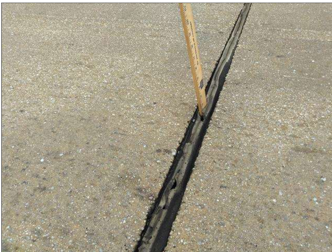
Span 83 Expansion Joint Bent 82: SCATTERED THROUGHOUT BOTH LANES, SEAL DAMAGE AND TORN (FULL WIDTH)
