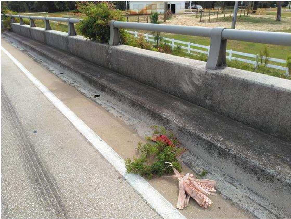
SPAN 247, RIGHT SHOULDER , 3RD SCUPPER CLOGGED BY VEGETATION AND OVERGROWTH OVER BARRIER THROUGHOUT
