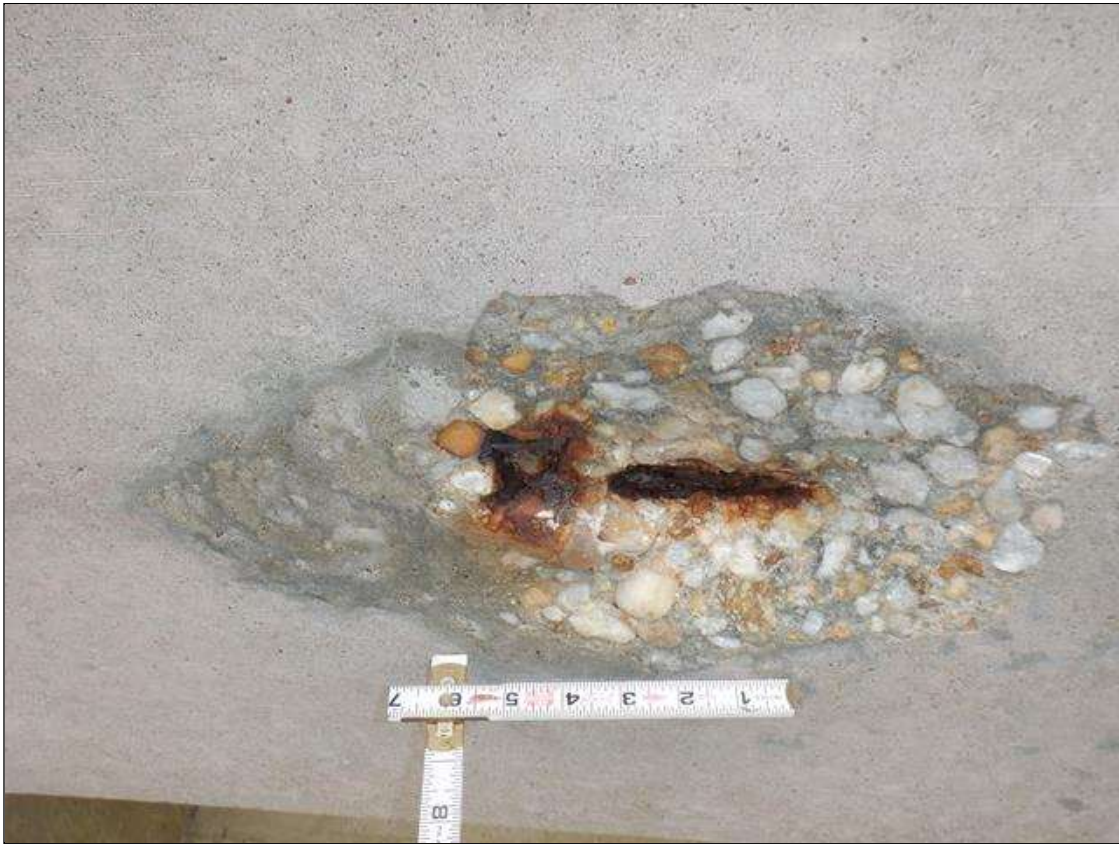
Span 92 Beam 3: (PAR) UNDERSIDE OF BOTTOM FLANGE AT 24 FEET FROM BENT 91, SPALL (9 INCHES X 8 INCHES X 1.5 INCHES) WITH EXPOSED STRAND (10 PERCENT SECTION LOSS)
