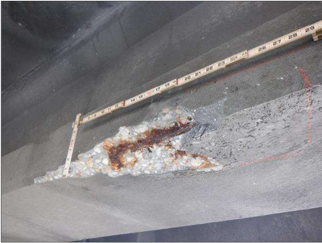
Span 124 Beam 2: (PAR) NORTH FACE OF BOTTOM FLANGE 10 FEET FROM BENT 124, UNSOUND PATCHED AREA (30 INCHES X 4 INCHES) WITH SPALL (16 INCHES X 5 INCHES X 2 INCHES X 1.5 INCHES DEEP) WITH (1) EXPOSED RUSTED STRAND (10 PERCENT SECTION LOSS)
