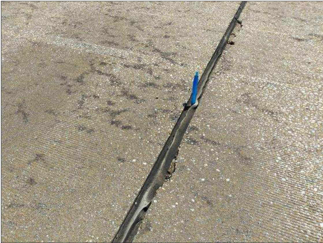
Span 172 Expansion Joint Bent 171: AT BENT 171, FULL WIDTH X FULL DEPTH WITH INTERMITTENT EDGE SPALLING UP TO 1 INCH WIDE
