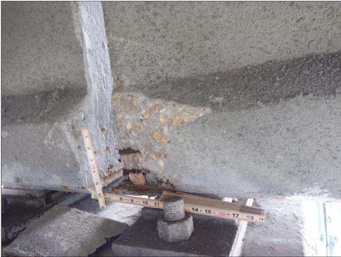
Span 135 Beam 4: (PAR) NORTH FACE OF BOTTOM FLANGE AT BENT 135, SPALL (10 INCHES X 9 INCHES X 2 INCHES) WITH (2) TWO EXPOSED STRANDS (10 PERCENT SECTION LOSS)
