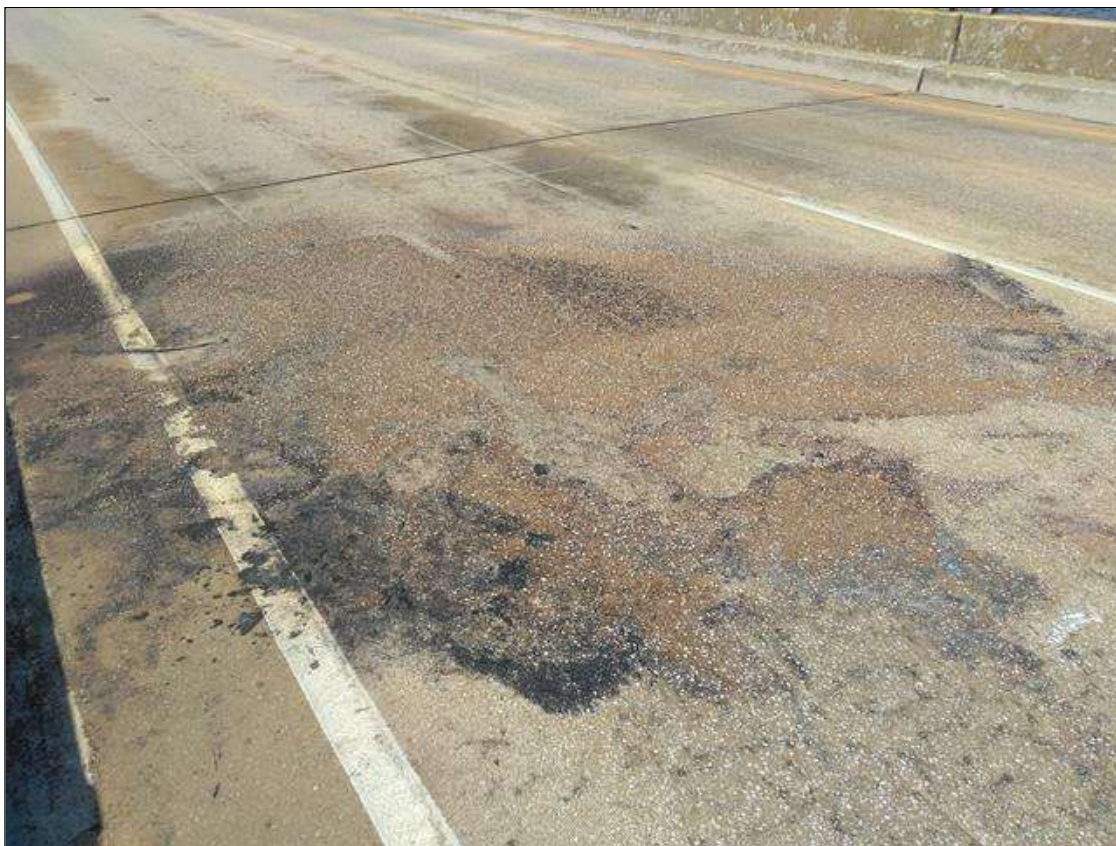
Span 148 Deck: STARTING AT BENT 147 IN RIGHT LANE, 13 FEET X 11 FEET X 0.25 INCHES SPALL (FIRE DAMAGE)
