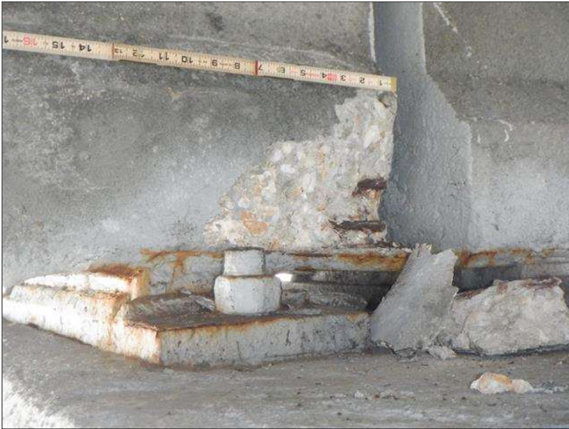
Span 101 Beam 3: (PAR) NORTH FACE OF BOTTOM FLANGE AT BENT 101, SPALL (11 INCHES LONG X 8 INCHES HIGH X 2 1/2 INCHES DEEP WITH (2) EXPOSED STRANDS (NO LOSS)
