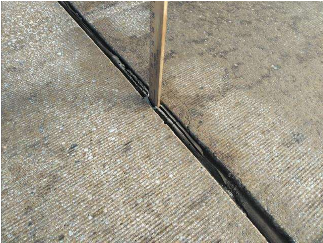
Span 205 Expansion Joint Bent 204: THROUGHOUT BOTH LANES, SEAL DAMAGED AND TORN FULL WIDTH X FULL DEPTH
