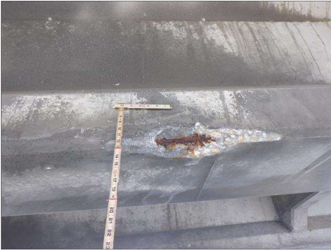
Span 130 Beam 3: (PAR) SOUTH FACE OF BOTTOM FLANGE AT 16 FEET FROM BENT 129, FAILED PATCH/SPALL (22 INCHES LONG X 3 INCHES HIGH X 4 INCHES WIDE X 1.5 INCHES DEEP) WITH (1) EXPOSED RUSTED STRAND (10 PERCENT SECTION LOSS)
