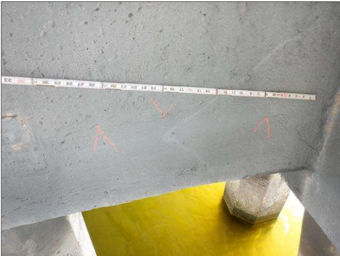
Bent 8 Cap 1: 1/32 INCHES TO 1/16 INCHES HORIZONTAL CRACK 2 FEET LONG ON WEST FACE OF CAP OVER PILE 4
