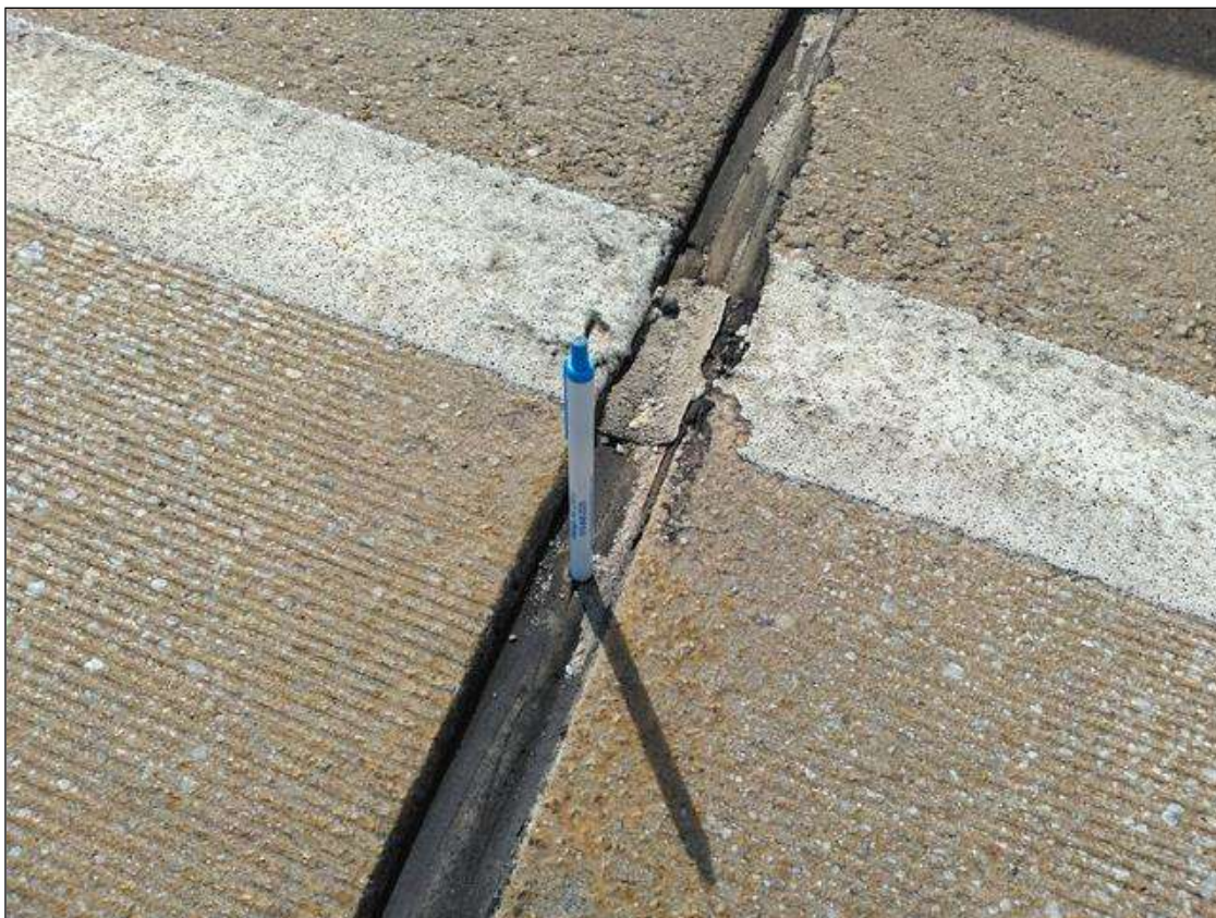
Span 225 Expansion Joint Bent 224: INTERMITTENT PARTIAL DEPTH CRACKING
