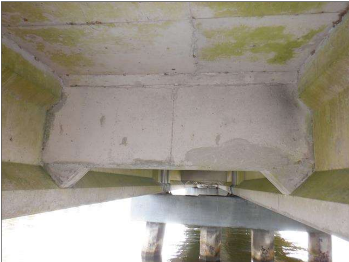
TYPICAL INTERIOR DIAPHRAGM
