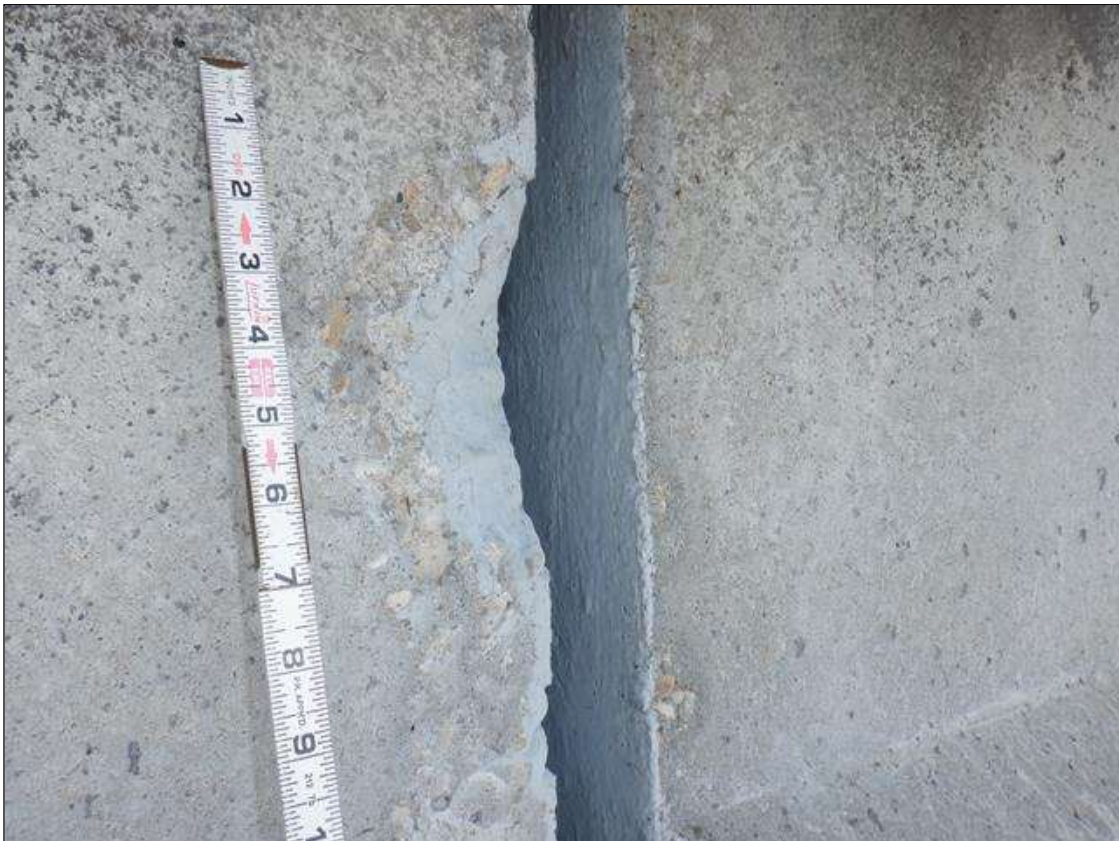
Span 35 Beam 4: SOUTH FACE OF BOTTOM FLANGE, AT BENT 35, SPALL (5 INCHES X 4 INCHES X 1 1/2 INCHES)
