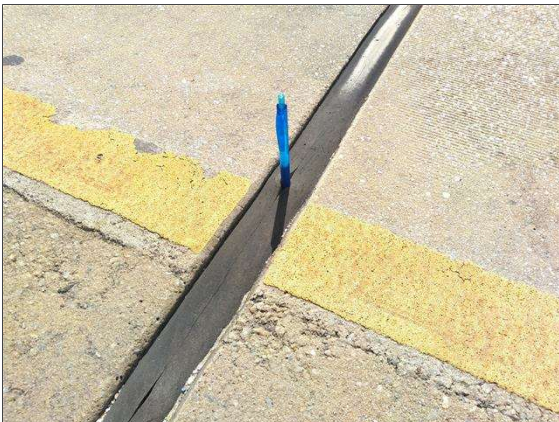
Span 140 Expansion Joint Bent 139: AT BENT 139, LEFT LANE 6 FOOT LONG PARTIAL DEPTH CRACK
