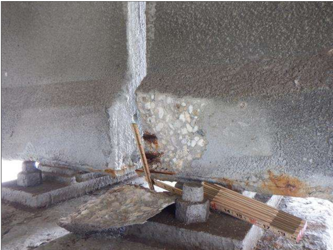
Span 126 Beam 4: (PAR) BOTTOM FLANGE NORTH FACE AT BENT 126, SPALL (6 INCHES X 6 INCHES X 2 INCHES DEEP) WITH (2) EXPOSED RUSTED STRANDS (NO LOSS)
