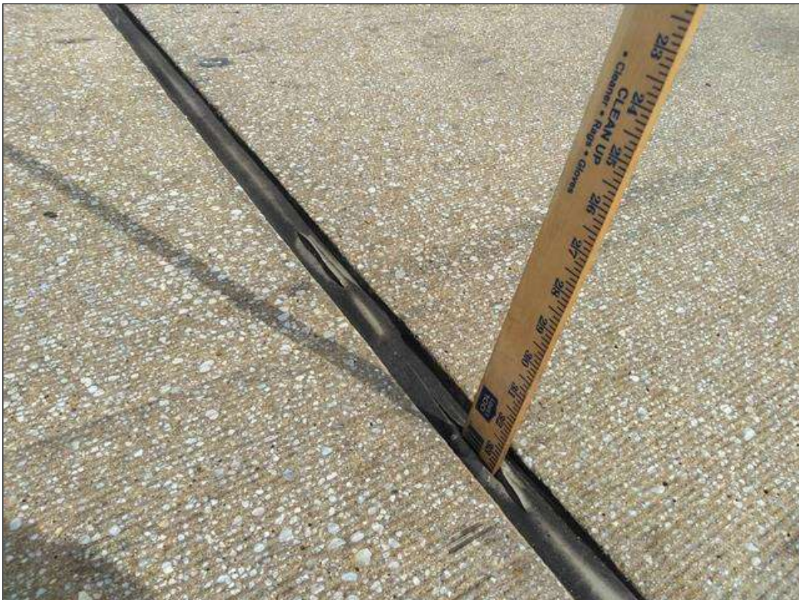
Span 240 Expansion Joint Bent 239: AT BENT 239, INTERMITTENT FULL DEPTH CRACKING THROUGHOUT
