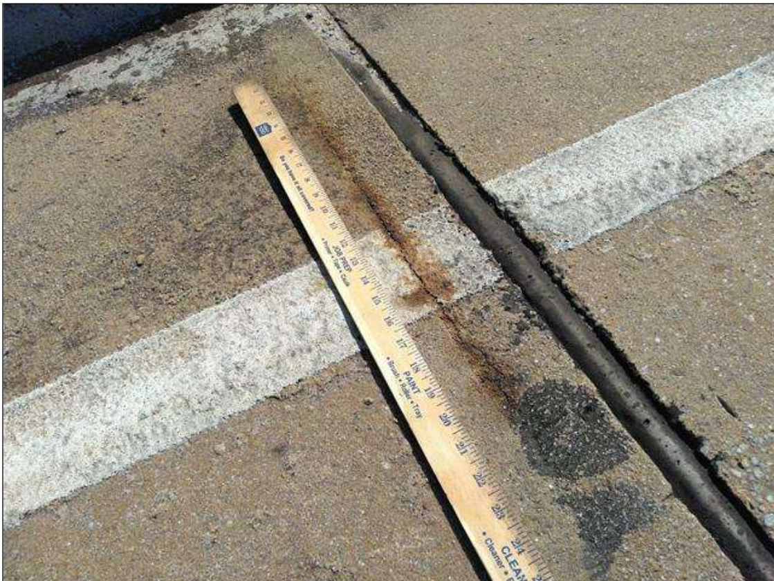
Span 200 Expansion Joint Bent 199: AT BENT 199, RIGHT LANE, PATCHED AREA ALONG JOINT WITH RUST STAINING
