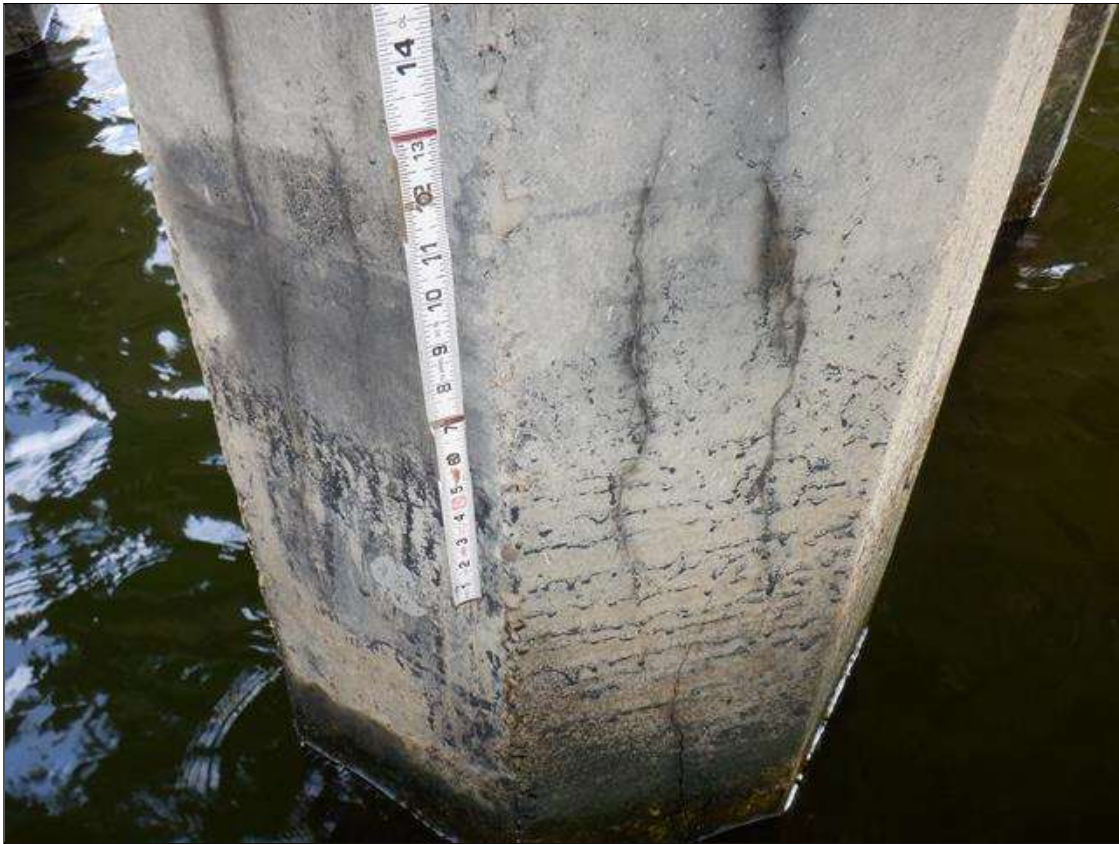
Bent 4 Pile 2: SCATTERED AROUND MULTIPLE FACES, VERTICAL CRACK (UP TO 4FEET X 1/32 INCHES)
