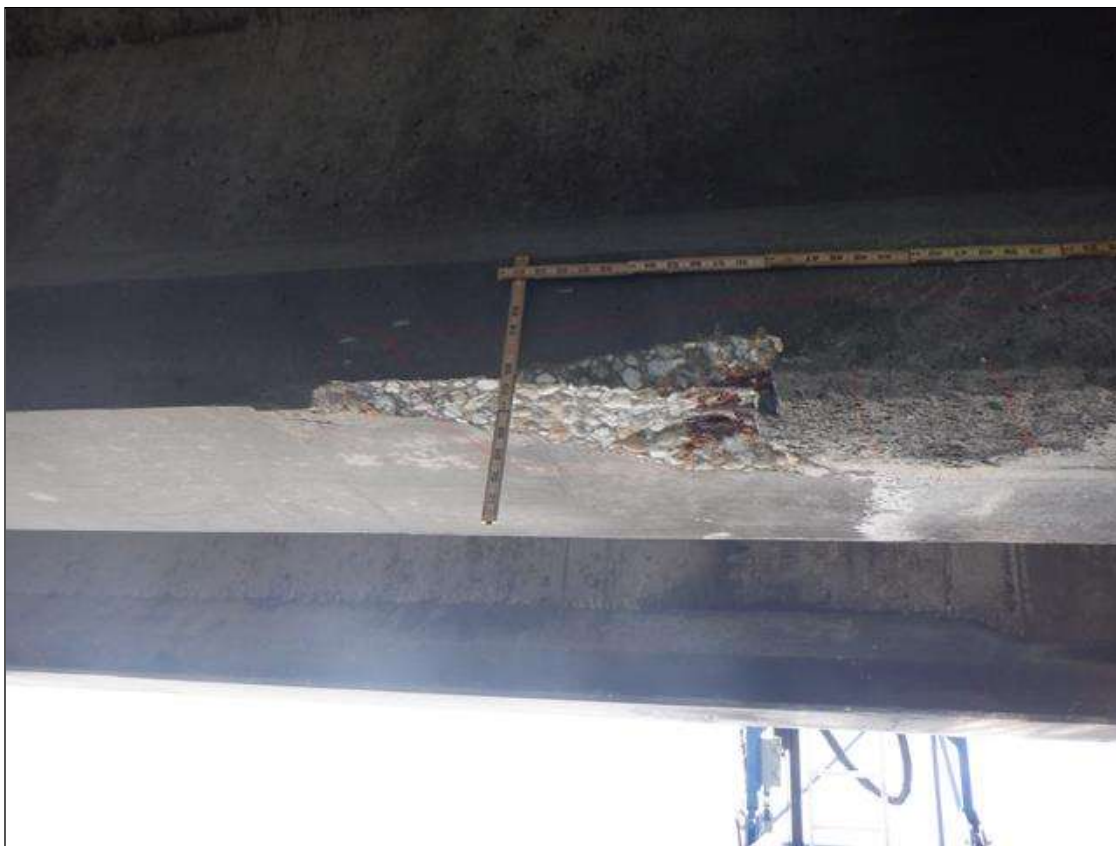
Span 104 Beam 3: UNDERSIDE OF BOTTOM FLANGE 6FEET FROM BENT 103, DELAMINATION/SPALL (48INCHES LONG X 5 INCHES HIGH X 11 INCHES ON BOTTOM X 1.5 INCHES DEEP) WITH (3) EXPOSED STRANDS (NO LOSS)
