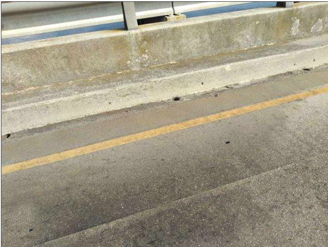
Span 2 Deck: DECK SURFACE 12 FEET FROM BENT 2 NEAR LEFT CURB, PATCHED AREA (12INCHES X 16 INCHES) (DEFECT NOT FOUND 9/12/22)
