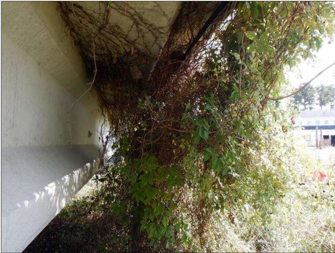
VEGETATION GROWING ON OVERHANGS AND EXTERIOR BEAMS
