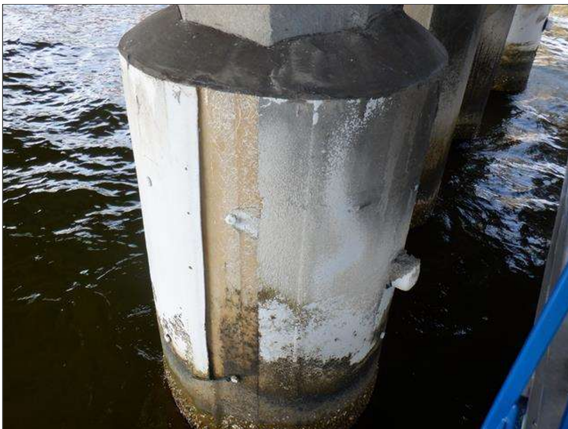
BENT 207 PILE 4: SOUTH FACE OF FIBERGLASS JACKET PARTIALLY BROKEN
