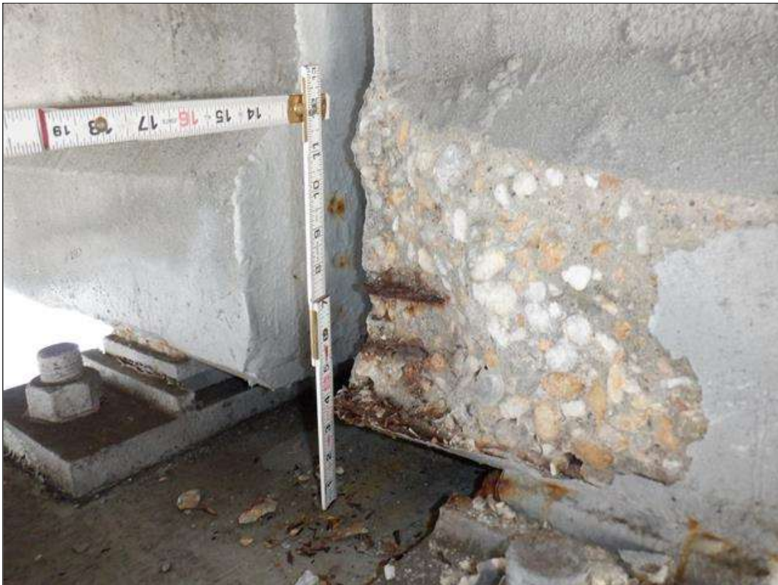
Span 76 Beam 2: (PAR) BOTTOM FLANGE SOUTH FACE AT BENT 75, SPALL (10 INCHES X 8 INCHES X 2 INCHES DEEP) WITH EXPOSED RUSTED STRANDS (10 PERCENT SECTION LOSS)
