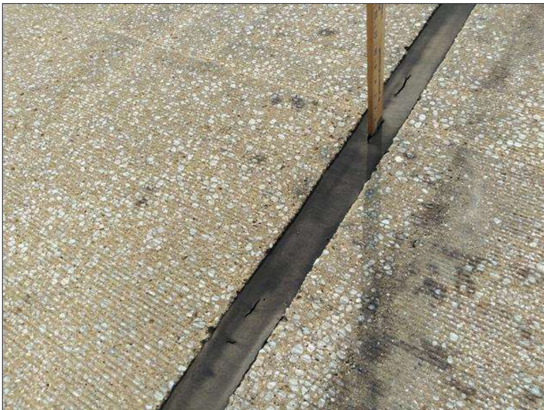
Span 248 Expansion Joint End Bent 2: AT END BENT 2, MULTIPLE FULL DEPTH CRACKS IN LEFT LANE
