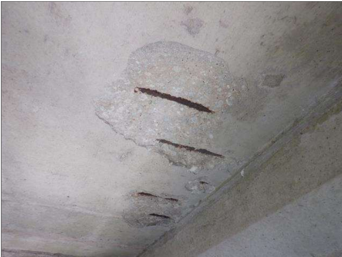
Span 181 Deck: UNDERSIDE OF DECK BAY 2 AT 4 FEET FROM BENT 181, SPALL (20 INCHES X 8 INCHES X 1 INCHES) WITH EXPOSED RUSTED REINFORCING
