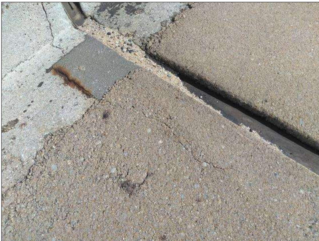
Span 223 Expansion Joint Bent 222: AT BENT 222, LEFT SHOULDER, DELAMINATION WITH RUST STAINING 2 FOOT X 4 INCH
