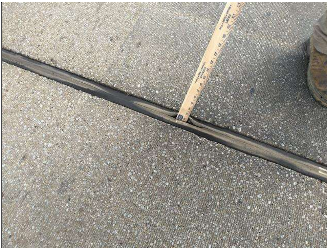
Span 3 Expansion Joint Bent 2: LEFT HALF SEAL DAMAGE
