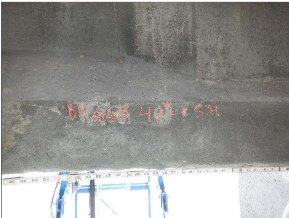
Span 68 Beam 4: NORTH FACE OF BOTTOM FLANGE AT BENT 67, SOUND PATCH (42 INCHES X 5 INCHES)
