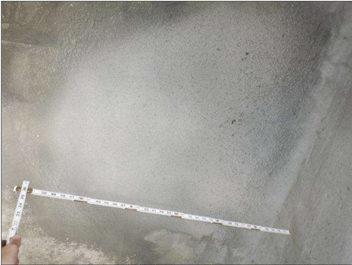
Span 6 Deck: UNDERSIDE OF DECK BAY 3 AT BENT 6, SOUND PATCH (3 FEET DIAMETER)
