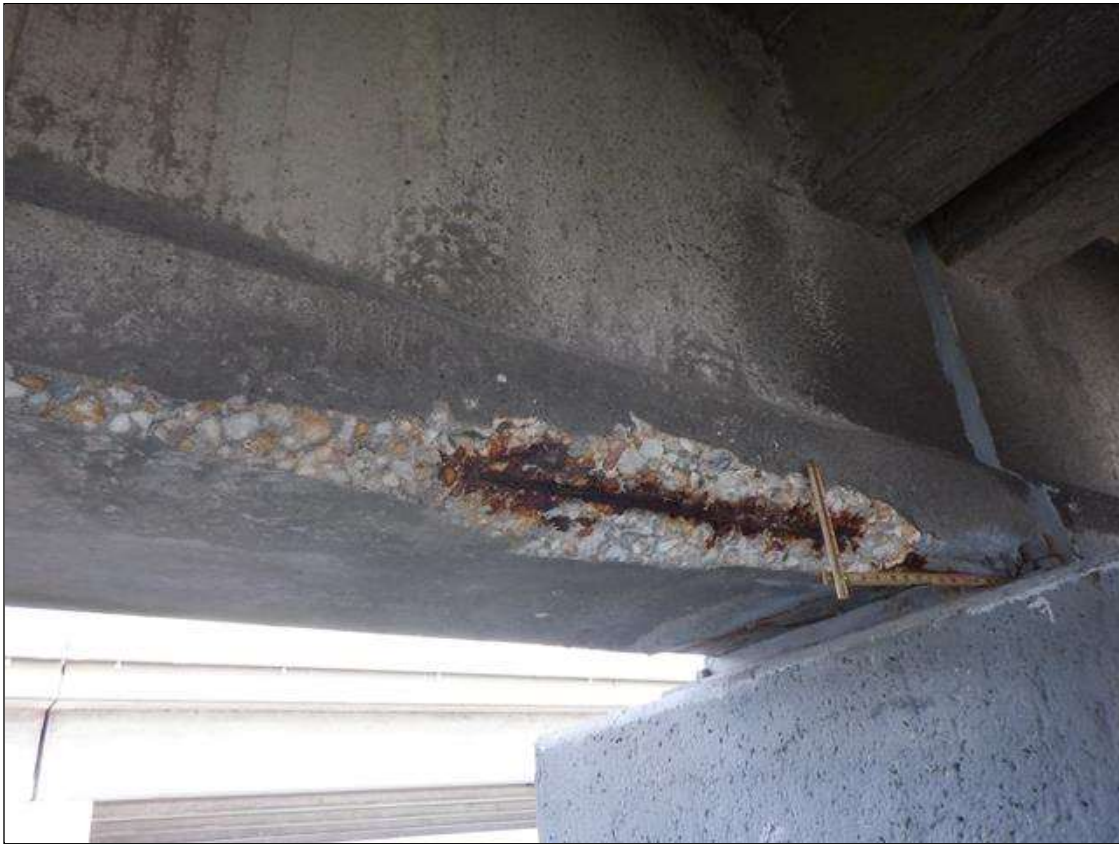
Span 126 Beam 1: (PAR) SOUTH FACE OF BOTTOM FLANGE AT 2 FEET FROM BENT 126, SPALL (48 INCHES LONG X 5 INCHES HIGH X 7 INCHES WIDE X 1.5 INCHES DEEP) WITH (1) ONE SEVERED STRAND
