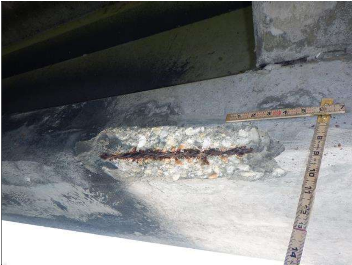
Span 231 Beam 4: (PAR) NORTH FACE OF BOTTOM FLANGE, AT 20 FEET FROM BENT 230, SPALL (18 INCHES X 5 INCHES X 2 INCHES) WITH EXPOSED STRAND (10 PERCENT SECTION LOSS) ON STRAND
