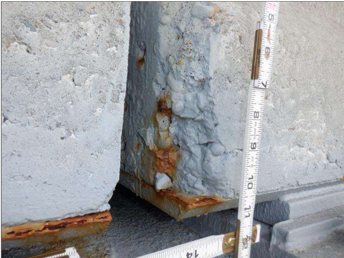
Span 67 Beam 1: NORTH FACE OF BOTTOM FLANGE , AT BENT 67, SPALL (3 INCHES X 6 INCHES X 2 INCHES) WITH EXPOSED STRANDS (NO SECTION LOSS)
