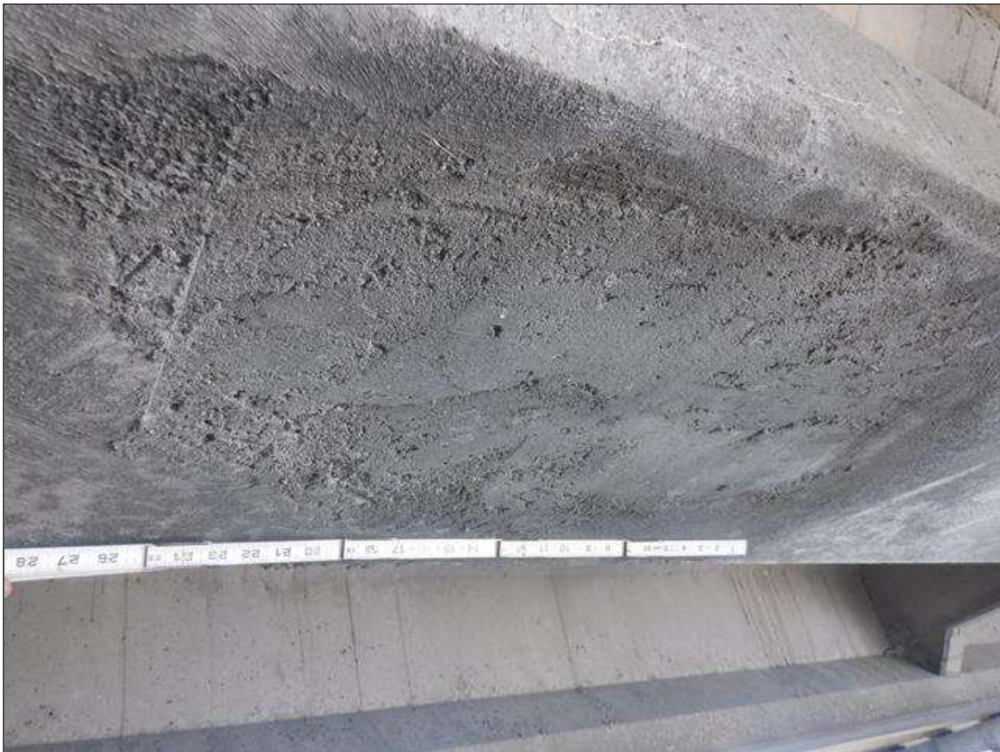
Span 98 Beam 2: UNDERSIDE OF BOTTOM FLANGE AT 6 FEET FROM BENT 97, UNSOUND PATCHED AREA (20 INCHES X 16 INCHES)
