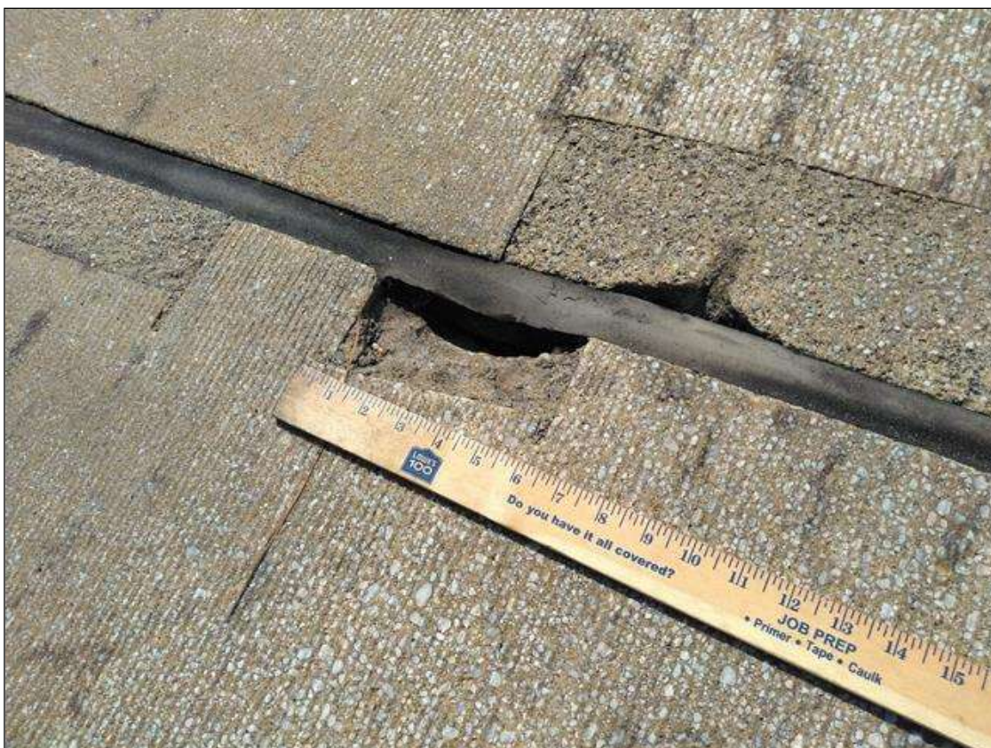
Span 188 Expansion Joint Bent 187: RIGHT RAIL ALONG JOINT, UNSOUND PATCHED AREAS (6INCHES X 3 INCHES)
