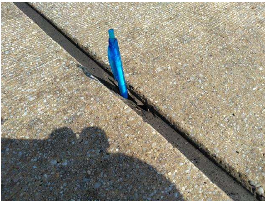
Span 147 Expansion Joint Bent 146: AT BENT 146, LEFT LANE, 4 INCH LONG PARTIAL DEPTH TEAR
