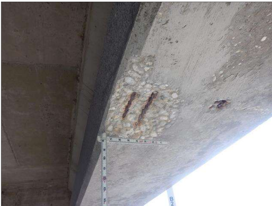
Span 184 Beam 4: (PAR) UNDERSIDE OF BOTTOM FLANGE AT MIDSPAN, SPALL (12 INCHES X 6 INCHES X 1 INCH) WITH TWO (2) EXPOSED STRANDS (15 PERCENT LOSS) ON STRANDS
