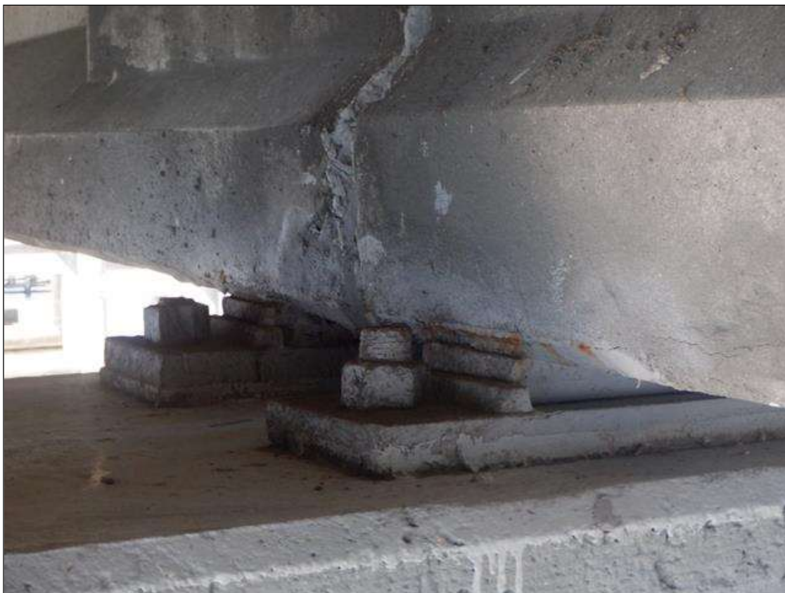
Span 187 Beam 1 - Far Bearing: MISSING ANCHOR BOLT NUT, SOUTH SIDE, AT BENT 187 - REPAIRED SINCE PREVIOUS INSPECTION 9/20/22
