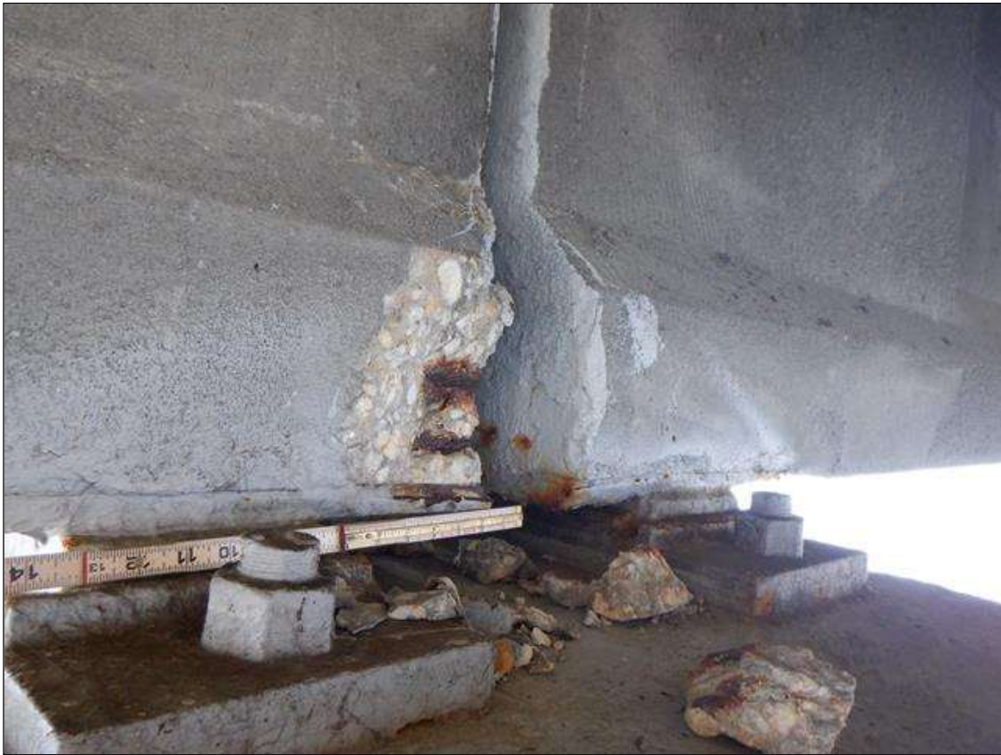
Span 215 Beam 3: (PAR) NORTH FACE OF BOTTOM FLANGE AT BENT 214, SPALL (7 INCHES X 7 INCHES X 2 INCHES) WITH (2) EXPOSED RUSTED STRANDS
