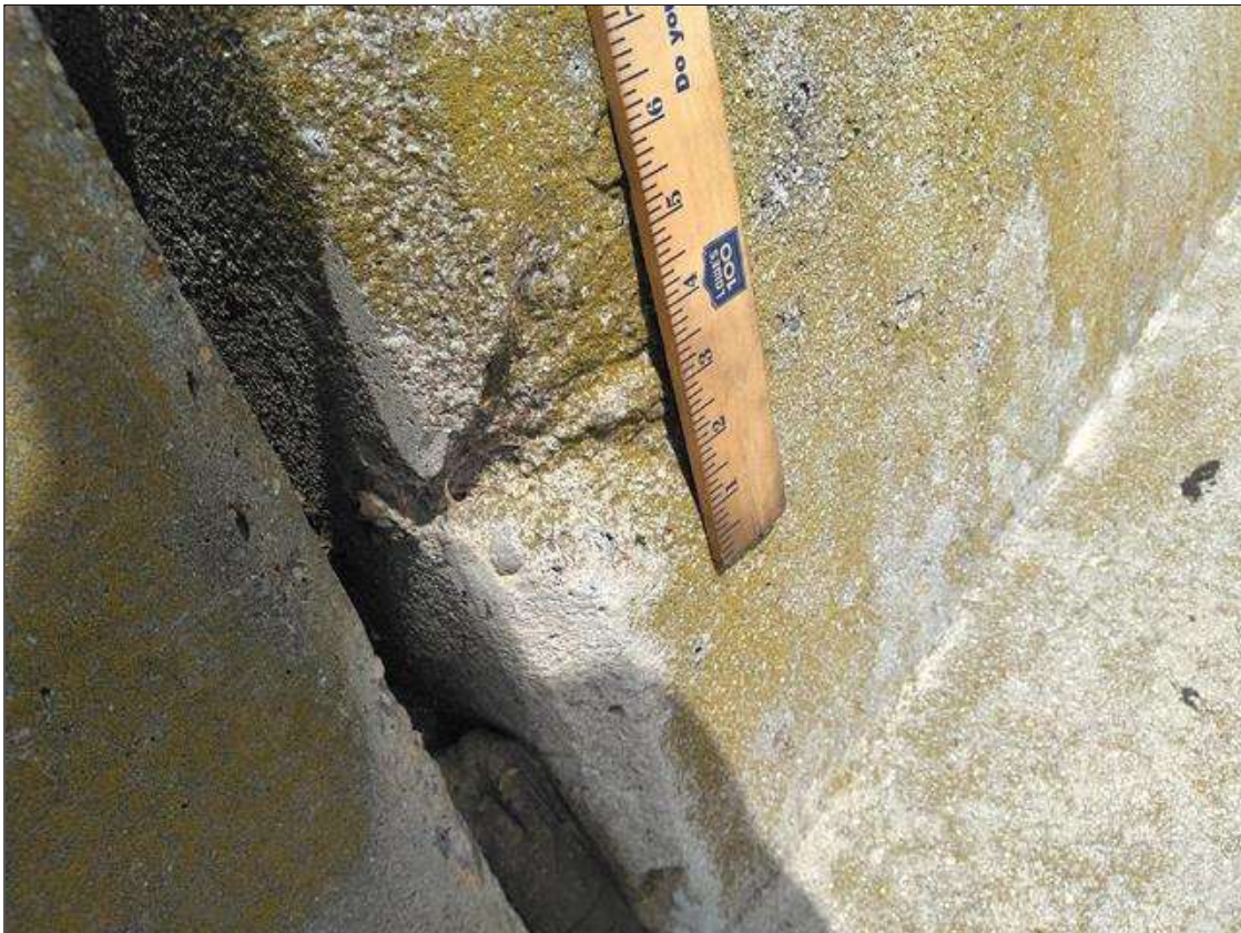
Span 155 Left Bridge Rail: AT BENT 154, SPALL 5 INCH DIAMETER X 1 INCH DEEP
