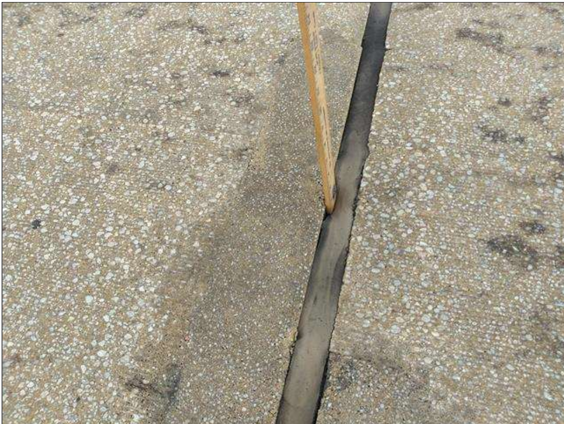
Span 72 Expansion Joint Bent 71: LEFT LANE NEAR CENTERLINE OF ROADWAY, (2) PATCHED AREAS (UP TO 1FEET X 5 INCHES). NO ADHESION AT PATCHES
