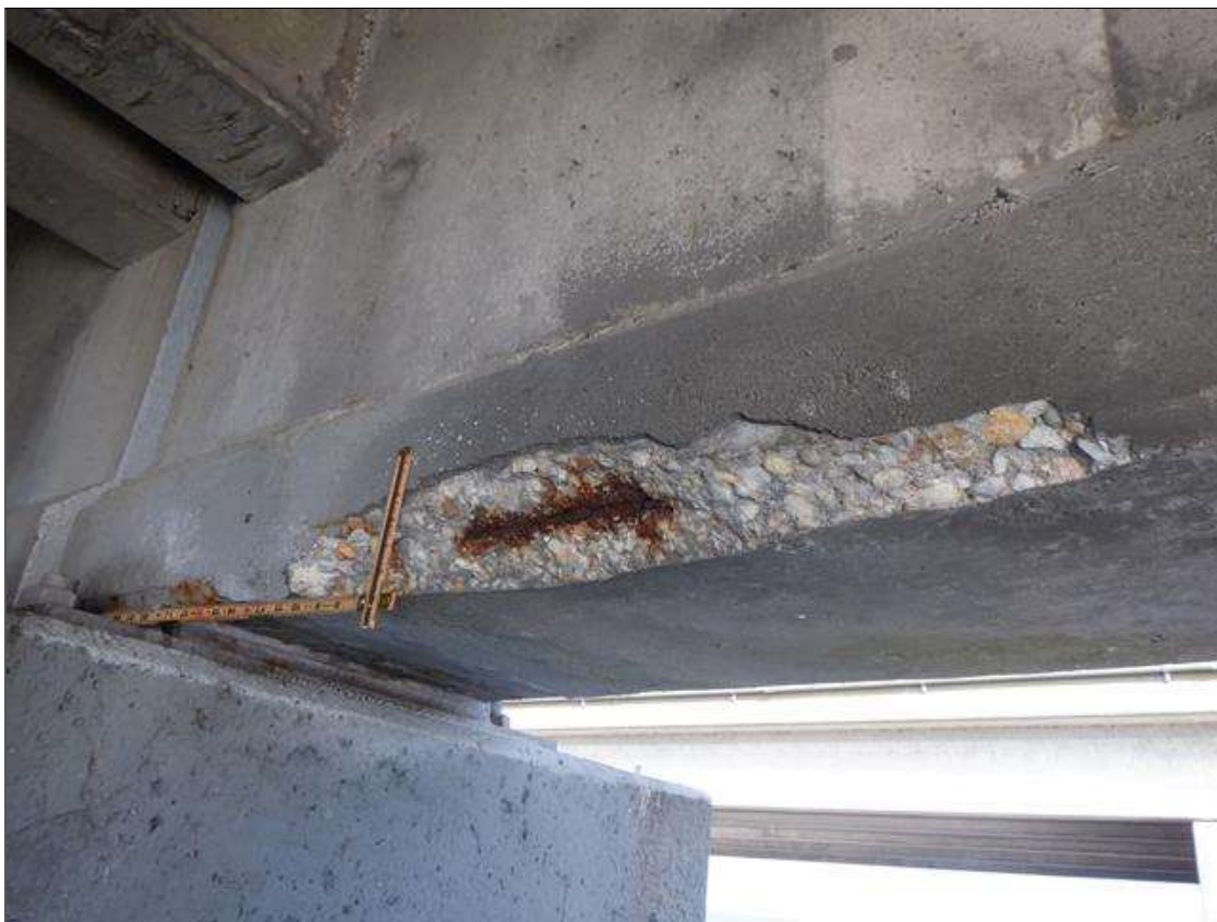
Span 119 Beam 1: (PAR) BOTTOM FLANGE SOUTH FACE AT BENT 118, SPALL (32 INCHES LONG X 4 INCHES HIGH X 3 INCHES WIDE X 2 INCHES DEEP) WITH (1) EXPOSED RUSTED STRAND (10 PERCENT SECTION LOSS)
