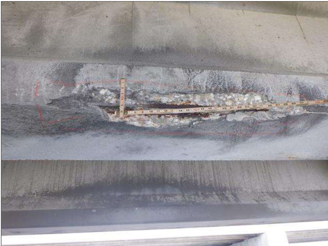
Span 104 Beam 2: (PAR) SOUTH FACE OF BOTTOM FLANGE NEAR MIDSPAN, SPALL (42 INCHES X 4 INCHES X 9 INCHES ON BOTTOM X 2 INCHES DEEP WITH (2) EXPOSED AND BROKEN STRANDS
