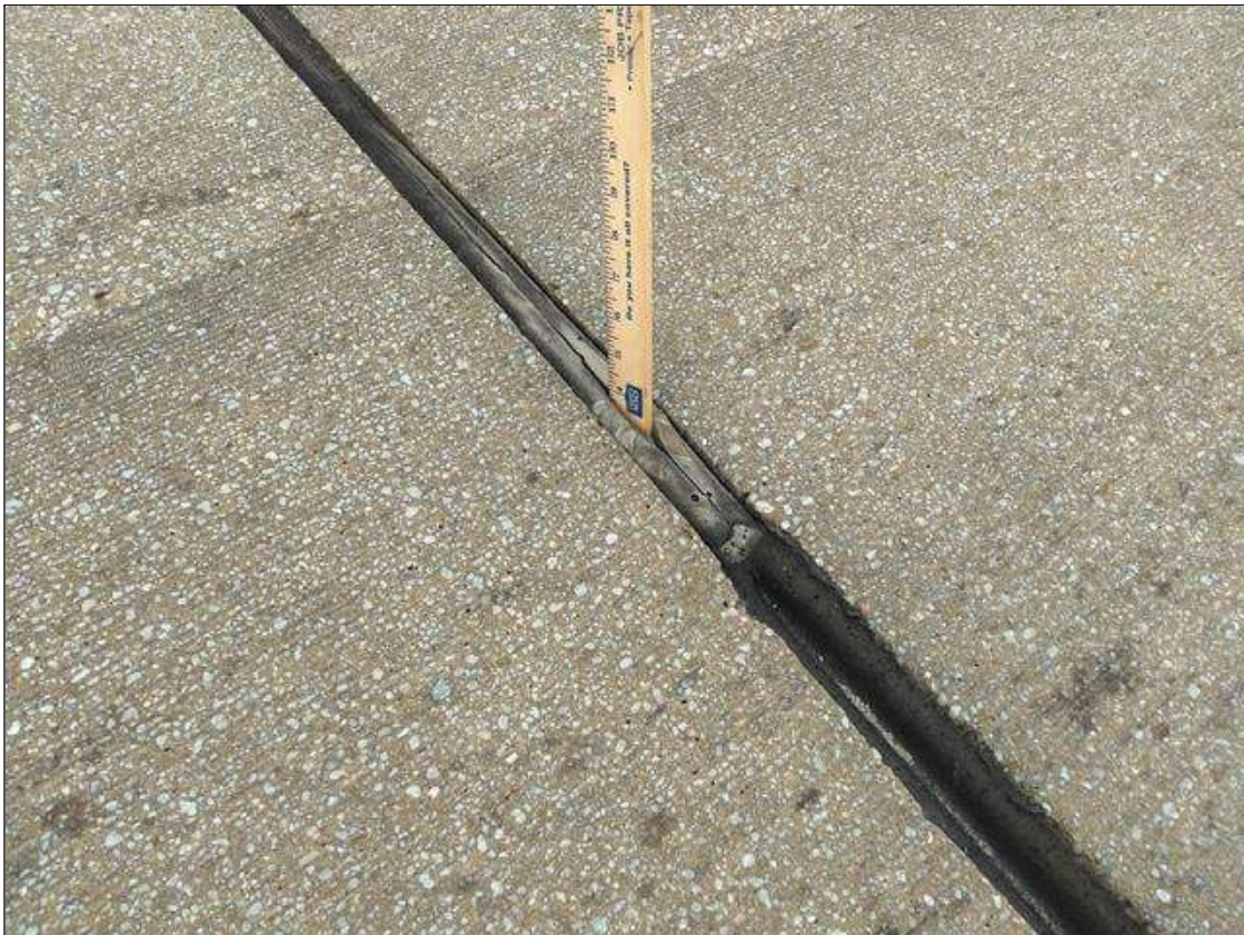
Span 95 Expansion Joint Bent 94: INTERMITTENT SPLITTING AND TEARING FULL DEPTCH IN LEFT SHOULDER TO CENTERLINE AND JOINT SUNKEN 1 INCH IN RIGHT LANE AND SHOULDER
