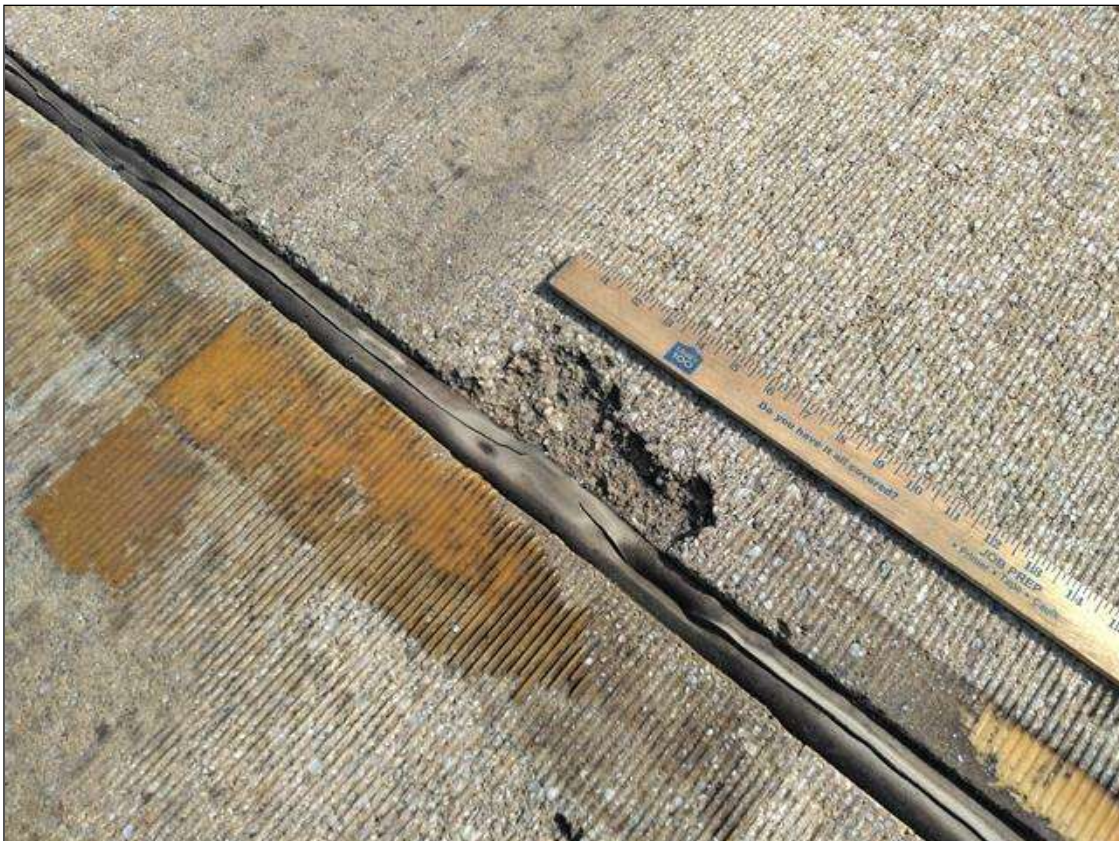
Span 119 Expansion Joint Bent 118: RIGHT LANE NEAR CENTERLINE OF ROADWAY, SPALL (6INCHES X 2INCHES X 1/2 INCHES)
