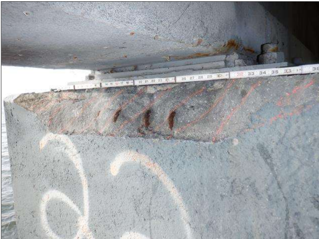
Bent 22 Cap 1: (PAR) TOP OF EAST FACE BELOW BEAM 4, SPALL (3.5 FEET X 6 INCHES 5 INCHES DEEP) WITH THREE (3) EXPOSED RUSTED REINFORCING (10 PERCENT SECTION LOSS)
