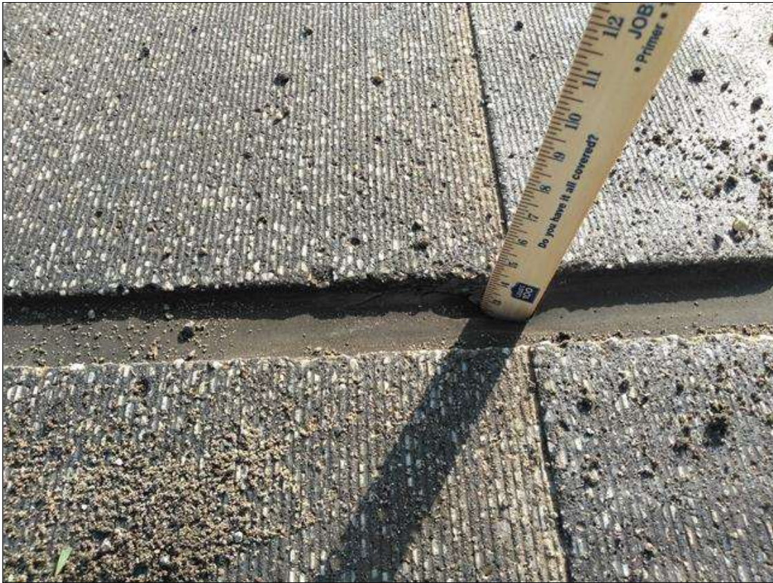
Span 1 Expansion Joint End Bent 1: AT END BENT 1 JOINT RIGHT EDGE OF TRAVEL, TEAR 6 INCH LONG X FULL DEPTH
