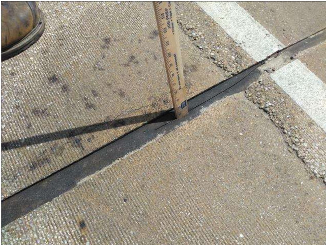
Span 47 Expansion Joint Bent 46: AT BENT 46, EACH SHOULDER 12 INCH LONG TEAR FULL DEPTH AND 24 INCH LONG TEAR FULL DEPTH AT CENTERLINE
