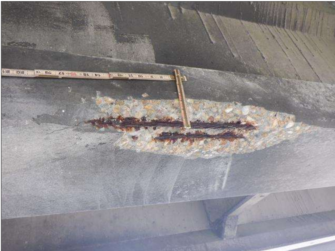
Span 137 Beam 2: (PAR) NORTH FACE OF BOTTOM FLANGE AT 16FEET FROM BENT 137, SPALL (27 INCHES X 8 INCHES X 2 INCHES) WITH (2) TWO EXPOSED STRANDS (20 PERCENT SECTION LOSS) ON STRAND
