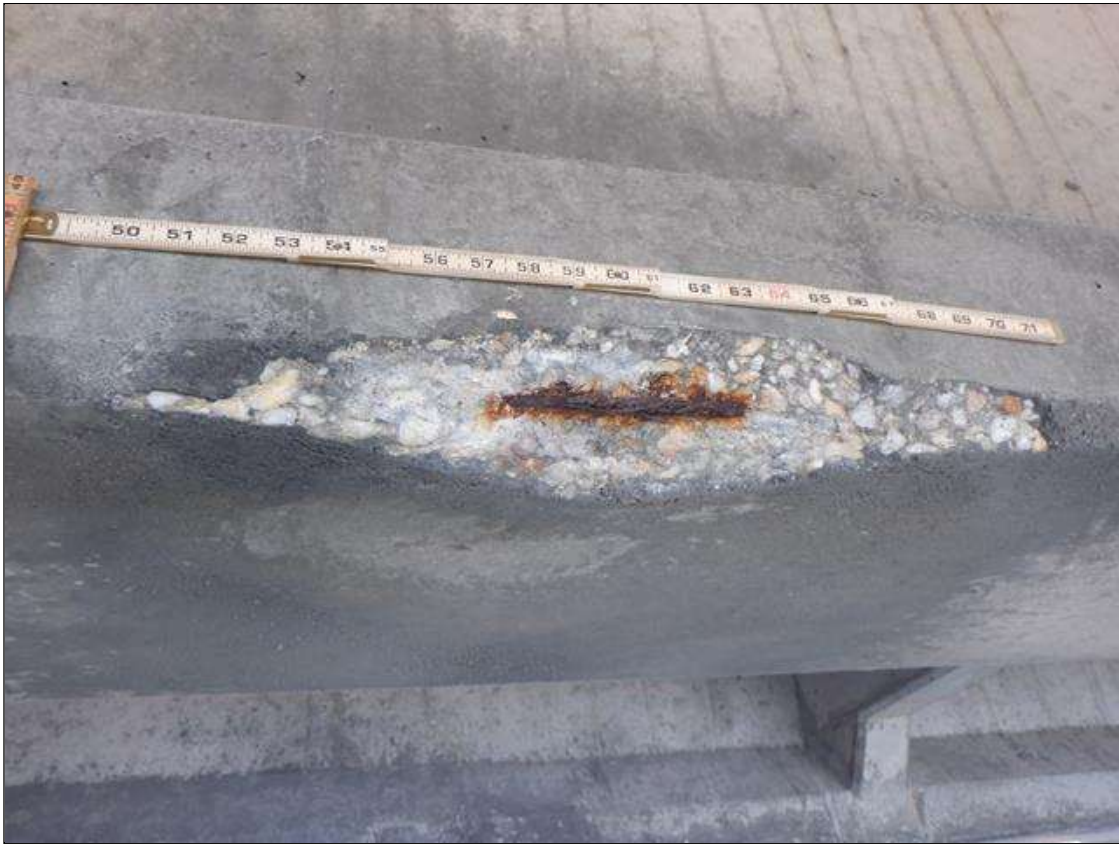
Span 224 Beam 2: (PAR) SOUTH FACE OF WEB, AT 16 FEET FROM BENT 223, SPALL (18 INCHES X 5 INCHES X 2 INCHES) WITH EXPOSED RUSTED STRAND (10 PERCENT SECTION LOSS) ON STRAND
