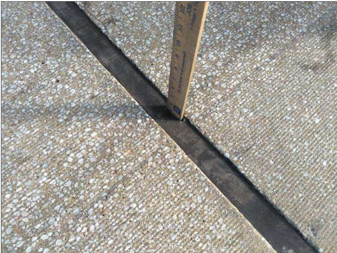
Span 209 Expansion Joint Bent 208: AT BENT 208, INTERMITTENT THROUGHOUT PARTIAL DEPTH CRACKING
