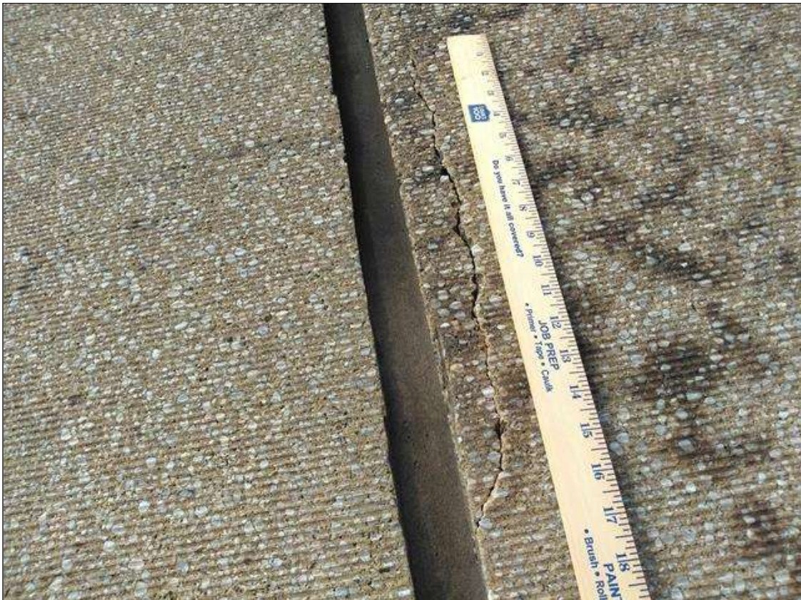
Span 16 Expansion Joint Bent 15: LEFT LANE, DELAMINATION 16 INCH WIDE X 2 INCH LONG
