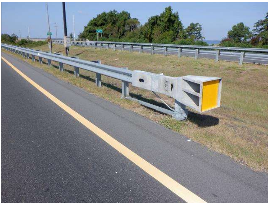
NORTHEAST GUARDRAIL END TREATMENT
