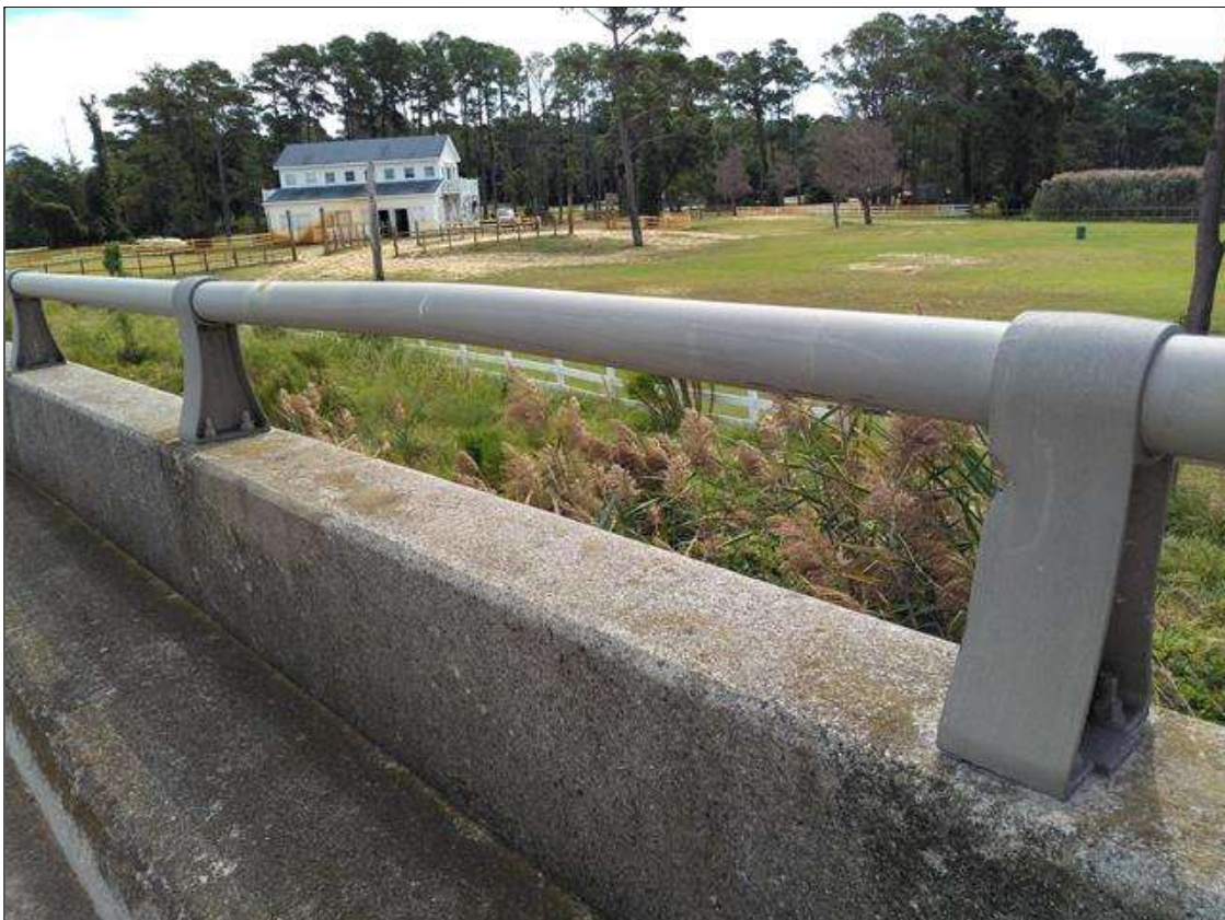
Span 245 Right Bridge Rail: POST 6, 2 INCH HIGH X 1 INCH LONG TEAR AND RAILING BETWEEN POSTS 6 AND 7 IS DEFLECTED 1 INCH AT MIDLENGTH
