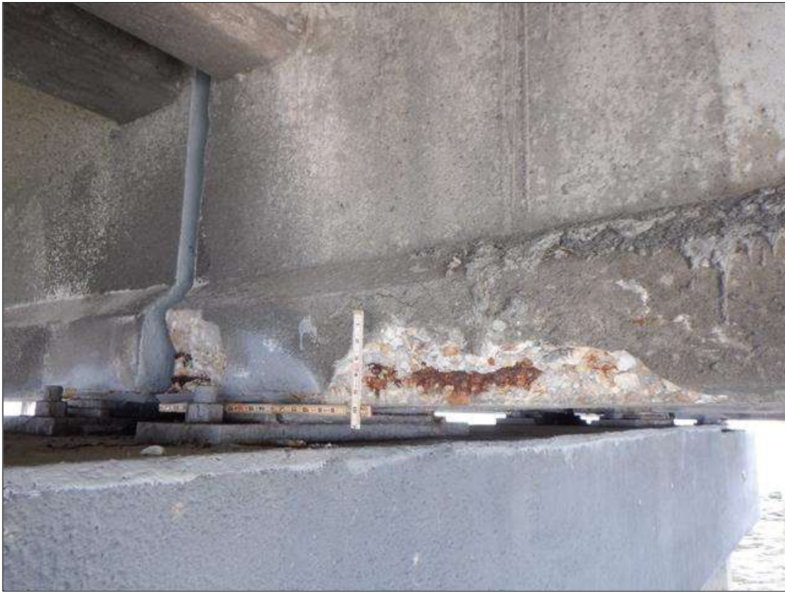
Span 127 Beam 3: (PAR) BOTTOM FLANGE SOUTH FACE AT BENT 126, (2) TWO SPALLS/DELAMINATIONS (UP TO 24 INCHES LONG X UP TO 8 INCHES HIGH X UP TO 2 INCHES DEEP) WITH (2) TWO EXPOSED RUSTED STRANDS (10 PERCENT SECTION LOSS)
