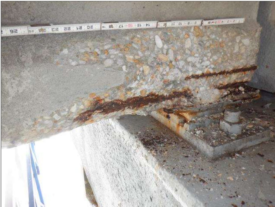
Span 87 Beam 3: (PAR) NORTH FACE OF BOTTOM FLANGE, AT BENT 86, SPALL (36 INCHES LONG X 9 INCHES HIGH X 2 INCHES DEEP) WITH TWO (2) EXPOSED RUSTED STRANDS (20 PERCENT SECTION LOSS)
