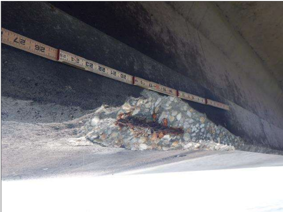
Span 224 Beam 4: (PAR) NORTH FACE OF BOTTOM FLANGE, AT 6 FEET FROM BENT 224, SPALL (30 INCHES X 8 INCHES X 2 INCHES) WITH EXPOSED STRANDS (10 PERCENT SECTION LOSS)
