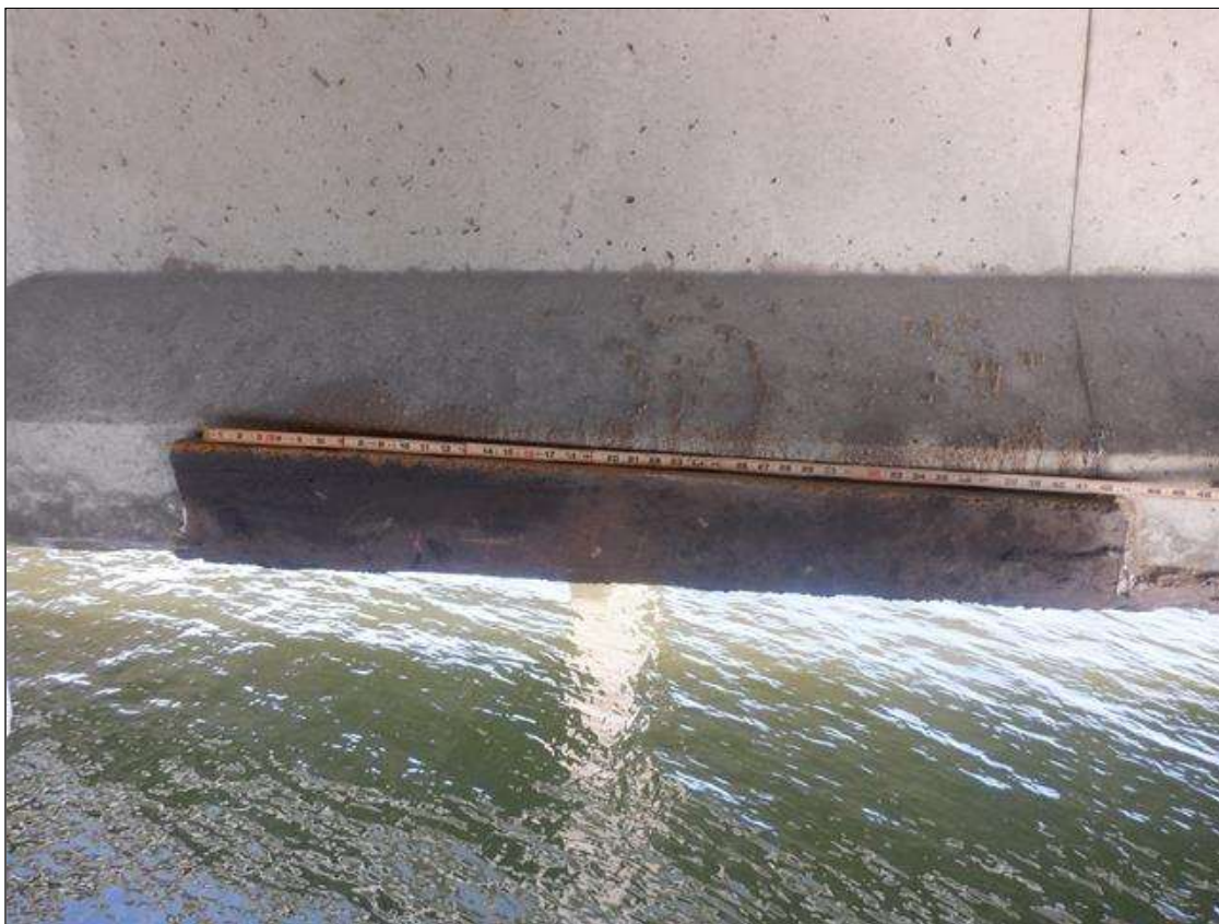
Span 165 Beam 1: BOTH FACES OF BOTTOM FLANGE AT 8 FEET FROM BENT 164, PATCHED AREA (48 INCHES X 7 INCHES)
