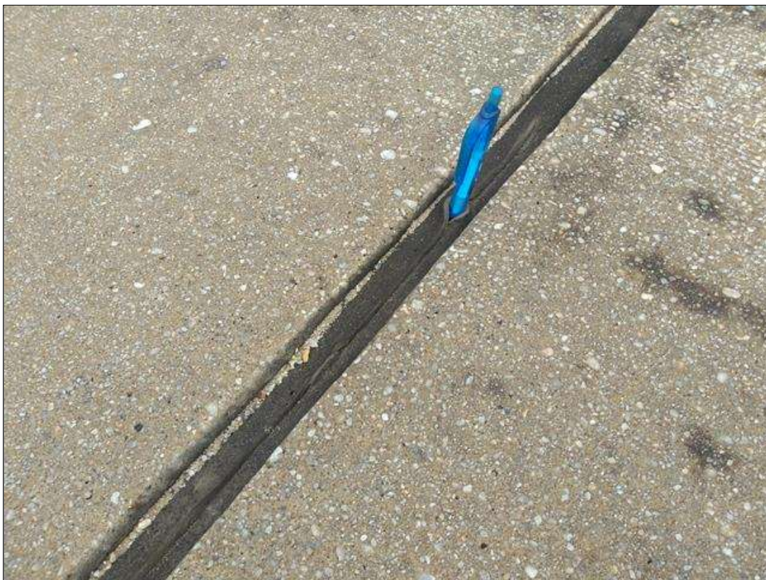
Span 107 Expansion Joint Bent 106: AT BENT 106, PARTIAL DEPTH TEAR INTERMITTENT THROUGH
