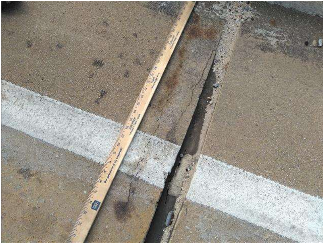
Span 202 Expansion Joint Bent 201: AT BENT 201, FULL DEPTH CRACKS AT BOTH SHOULDERS AND CENTERLINE
