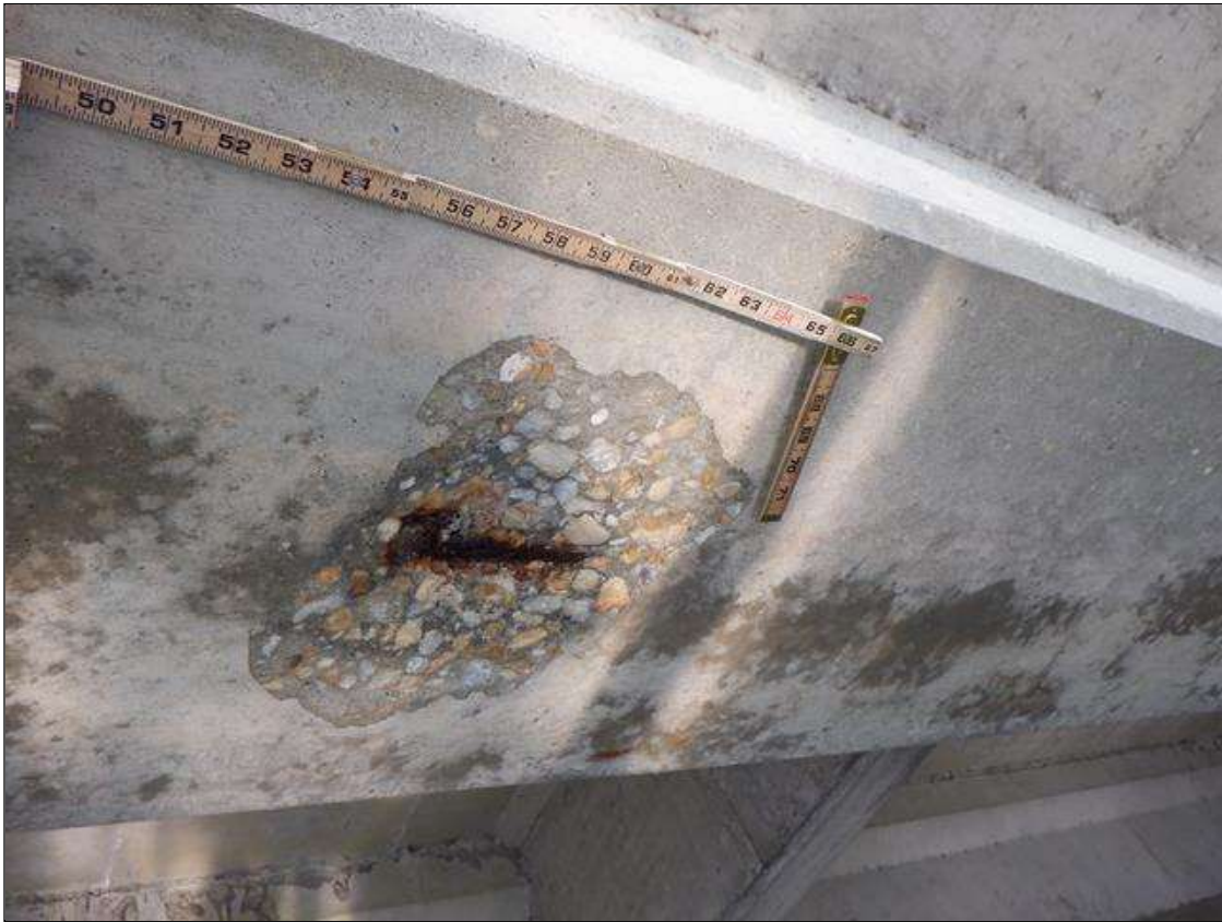
Span 148 Beam 4: (PAR) UNDERSIDE OF BOTTOM FLANGE AT 24FEET FROM BENT 148, SPALL (12INCHES DIAMETER X 1 INCHES) WITH EXPOSED STRANDS (5 PERCENT SECTION LOSS) ON STRAND
