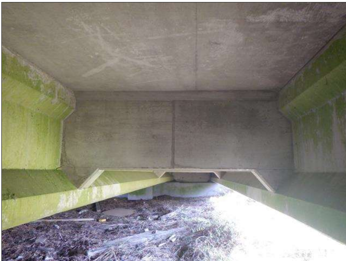
TYPICAL INTERIOR DIAPHRAGM
