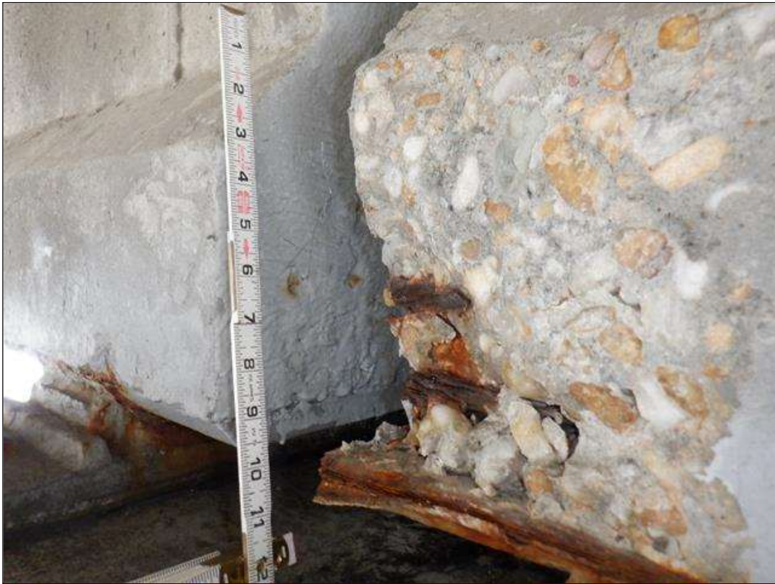
Span 82 Beam 3: (PAR) NORTH FACE OF BOTTOM FLANGE, AT BENT 82, SPALL (7INCHES X 9INCHES X 2 INCHES) WITH EXPOSED STRANDS (10 PERCENT SECTION LOSS)
