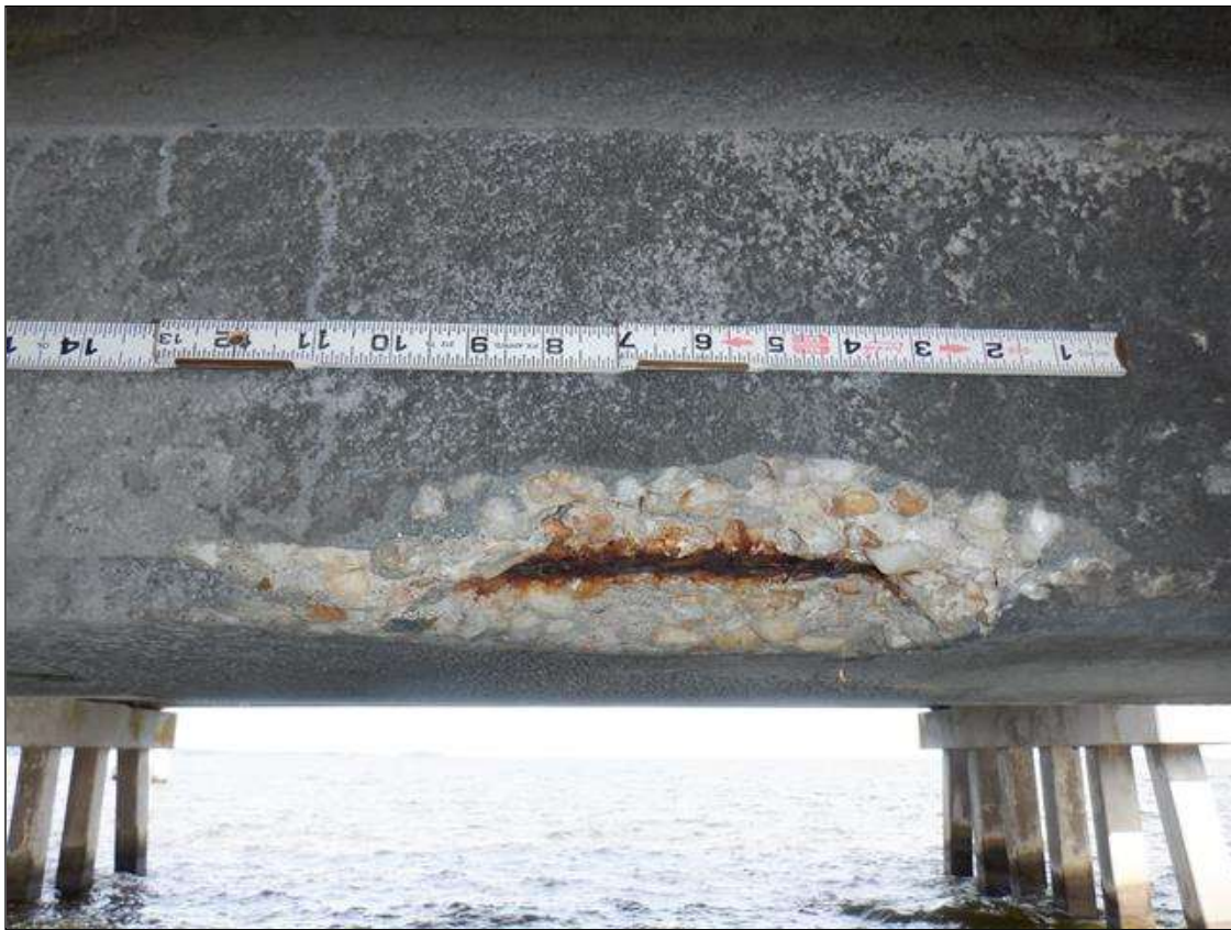
Span 58 Beam 1: (PAR) SOUTH FACE OF BOTTOM FLANGE, AT 22 FEET FROM BENT 58, FAILED PATCH/SPALL (12 INCHES X 5 INCHES X 2 INCHES) WITH EXPOSED RUSTED STRAND, SECTION LOSS (10 PERCENT)
