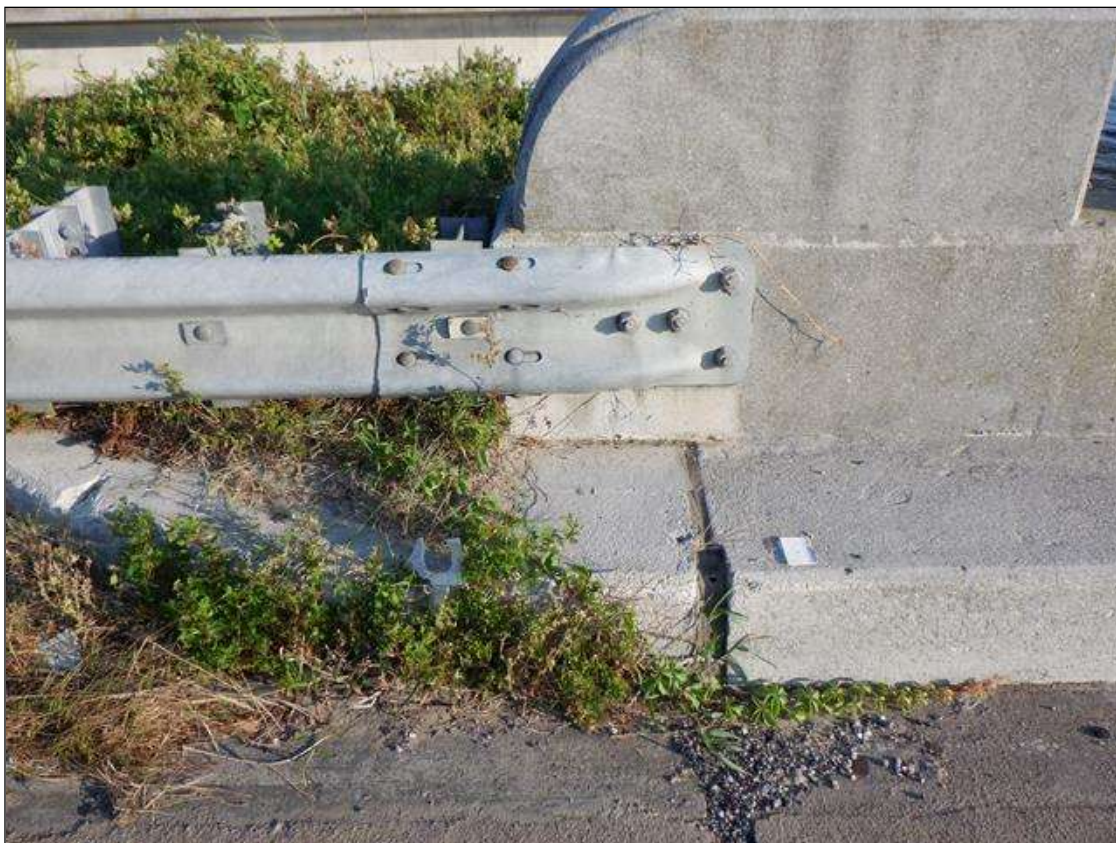
TYPICAL GUARDRAIL ATTACHMENT, NORTHWEST IN VIEW
