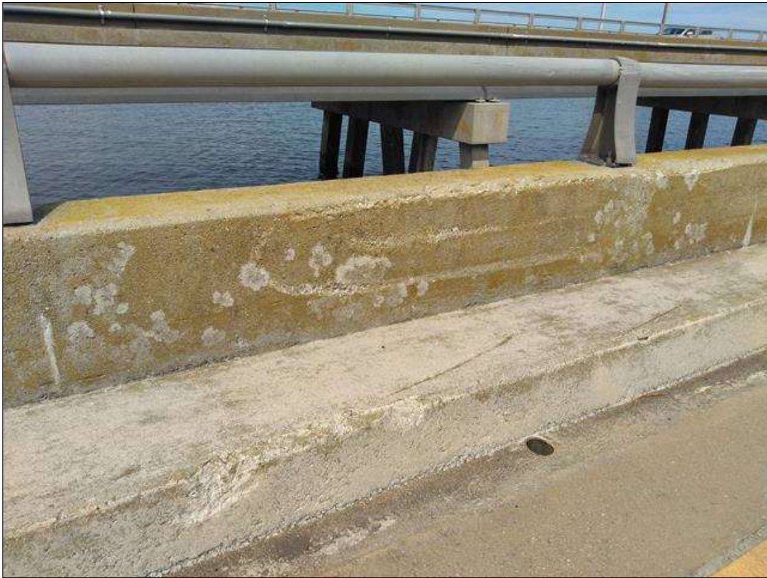
Span 68 Left Bridge Rail: (PAR) RAILPOSTS 4 TO 7, IMPACT SCRAPES (UP TO 20 FEET)
