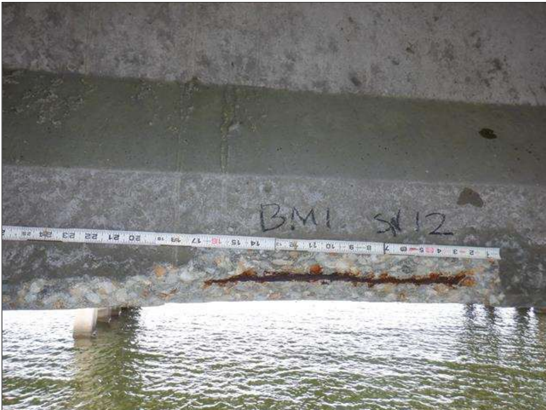
Span 12 Beam 1: (PAR) BOTTOM FLANGE SOUTH FACE, 12 FEET FROM BENT 11, SPALL (24 INCHES X 4 INCHES X 3 INCHES DEEP) WITH EXPOSED RUSTED STRANDS (25 PERCENT SECTION LOSS)
