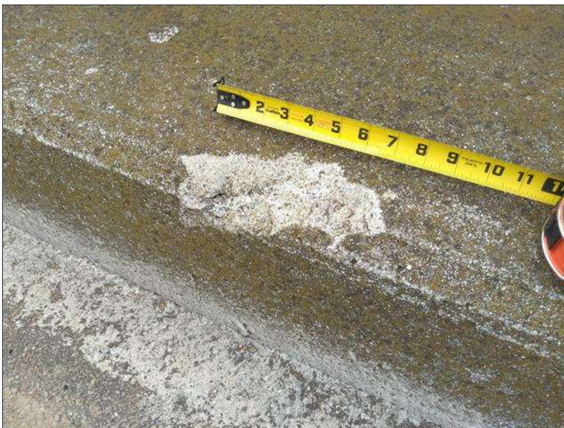
Span 105 Right Bridge Rail: CURB BETWEEN POSTS 6 AND 7, SPALL (8INCHES X 3INCHES X 1 INCHES)
