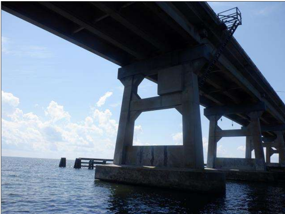
TYPICAL INTERIOR BENT PROFILE, TWO PILES WITH HAUNCH IN VIEW
