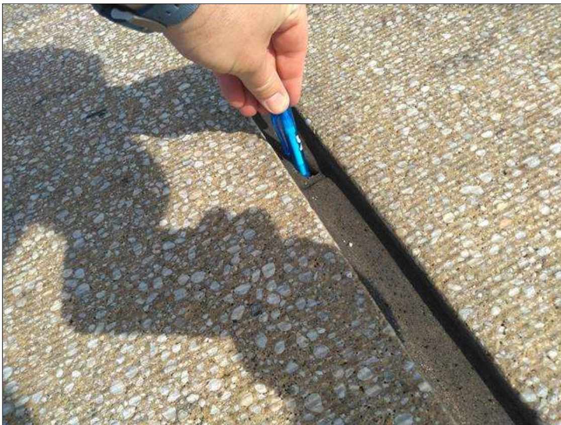
Span 132 Expansion Joint Bent 131: AT BENT 131, 2 INCH WIDE X FULL DEPTH CRACK IN RIGHT LANE
