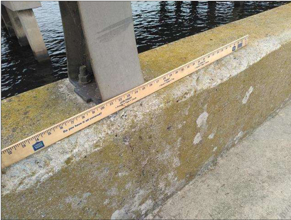
Span 82 Left Bridge Rail: RAILPOST 8, IMPACT SPALL (4FEET X 6INCHES X 1/2 INCHES)
