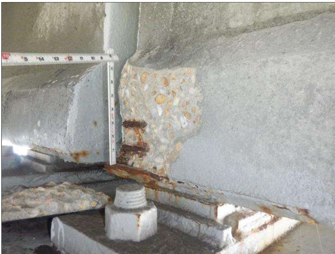
Span 198 Beam 2: (PAR) NORTH FACE OF BOTTOM FLANGE AT BENT 198, SPALL (9 INCHES X 9 INCHES X 2 1/2 INCHES DEEP) WITH TWO (2) EXPOSED STRANDS (10 PERCENT LOSS)
