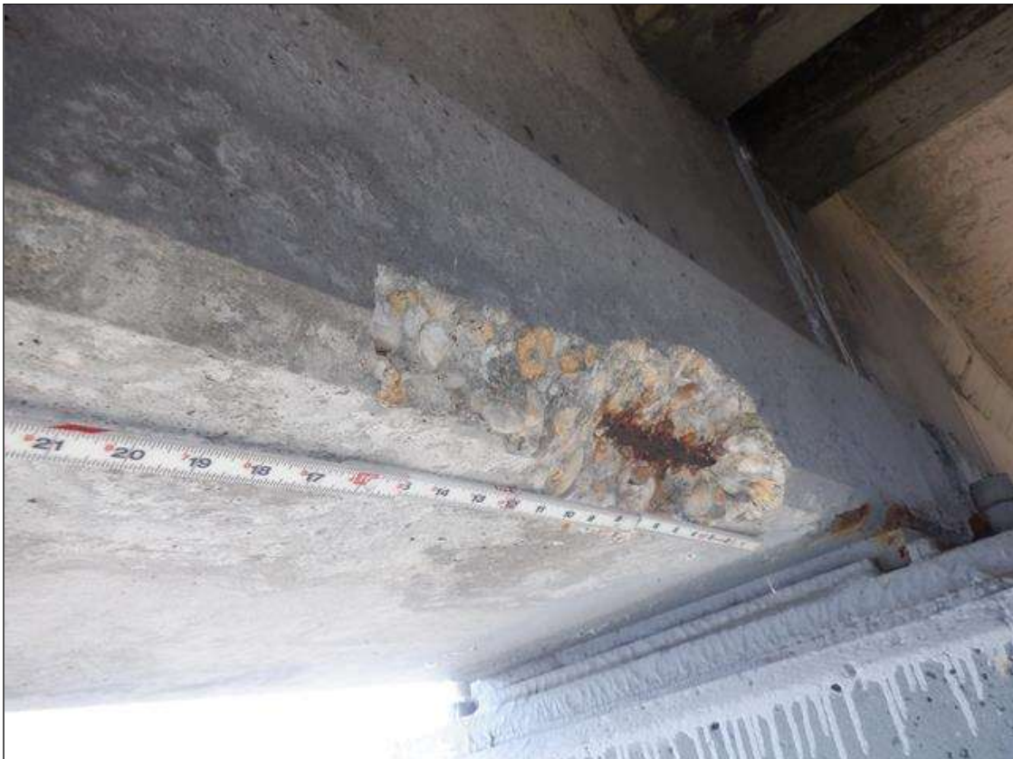
Span 174 Beam 4: (PAR) NORTH FACE 2 FEET EAST OF BENT 173, SPALL (1 1/2 FEET X 3 INCHES X 2 INCHES DEEP) WITH ONE (1) EXPOSED STARND (10 PERCENT LOSS)
