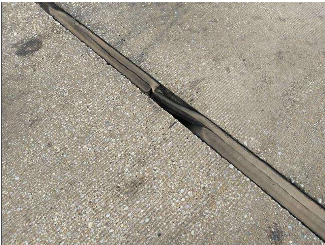
Span 3 Expansion Joint Bent 2: RIGHT HALF, SEAL DAMAGE
