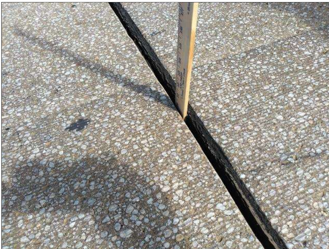
Span 36 Expansion Joint Bent 35: BOTH LANES AND SHOULDERS, SEAL DAMAGE (FULL DEPTH X FULL LENGTH)
