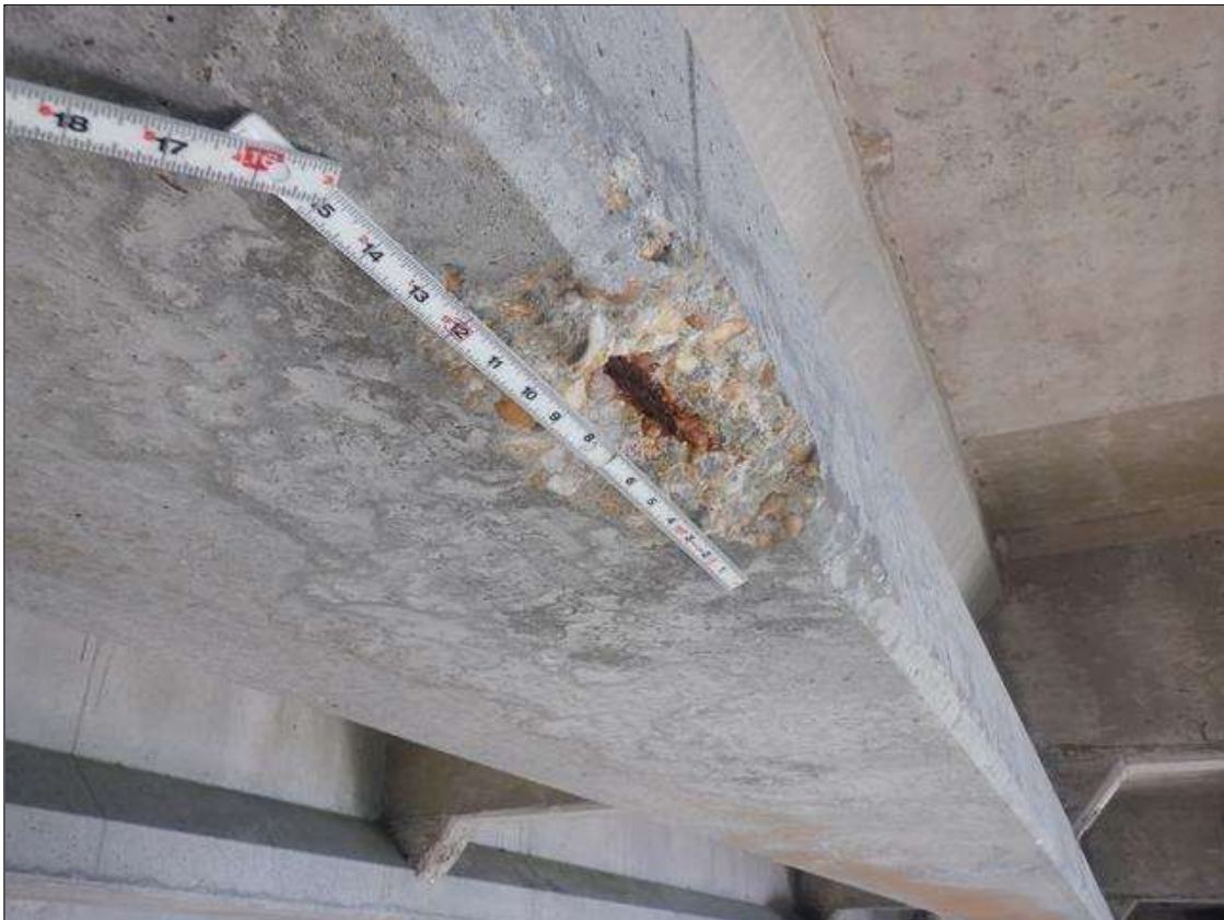
Span 186 Beam 3: (PAR) SOUTH FACE OF BOTTOM FLANGE AT 10 FEET FROM BENT 185, SPALL (1 FOOT X 4 INCHES X 1 1/2 INCHES DEEP)
