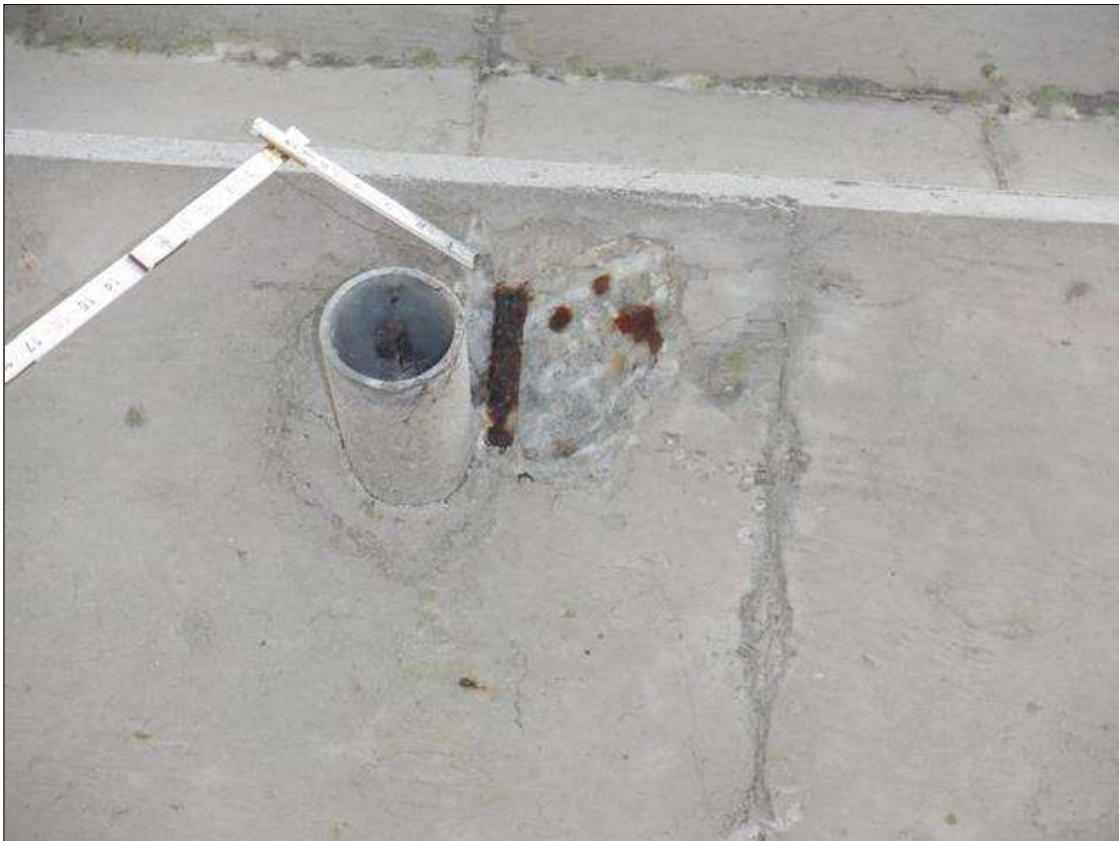
Span 18 Deck: UNDERSIDE LEFT OVERHANG NEAR MIDSPAN, TWO (2) SPALLS (6 INCH DIAMETER X 2 INCHES DEEP) WITH EXPOSED RUSTED REINFORCING (10 PERCENT SECTION LOSS)
