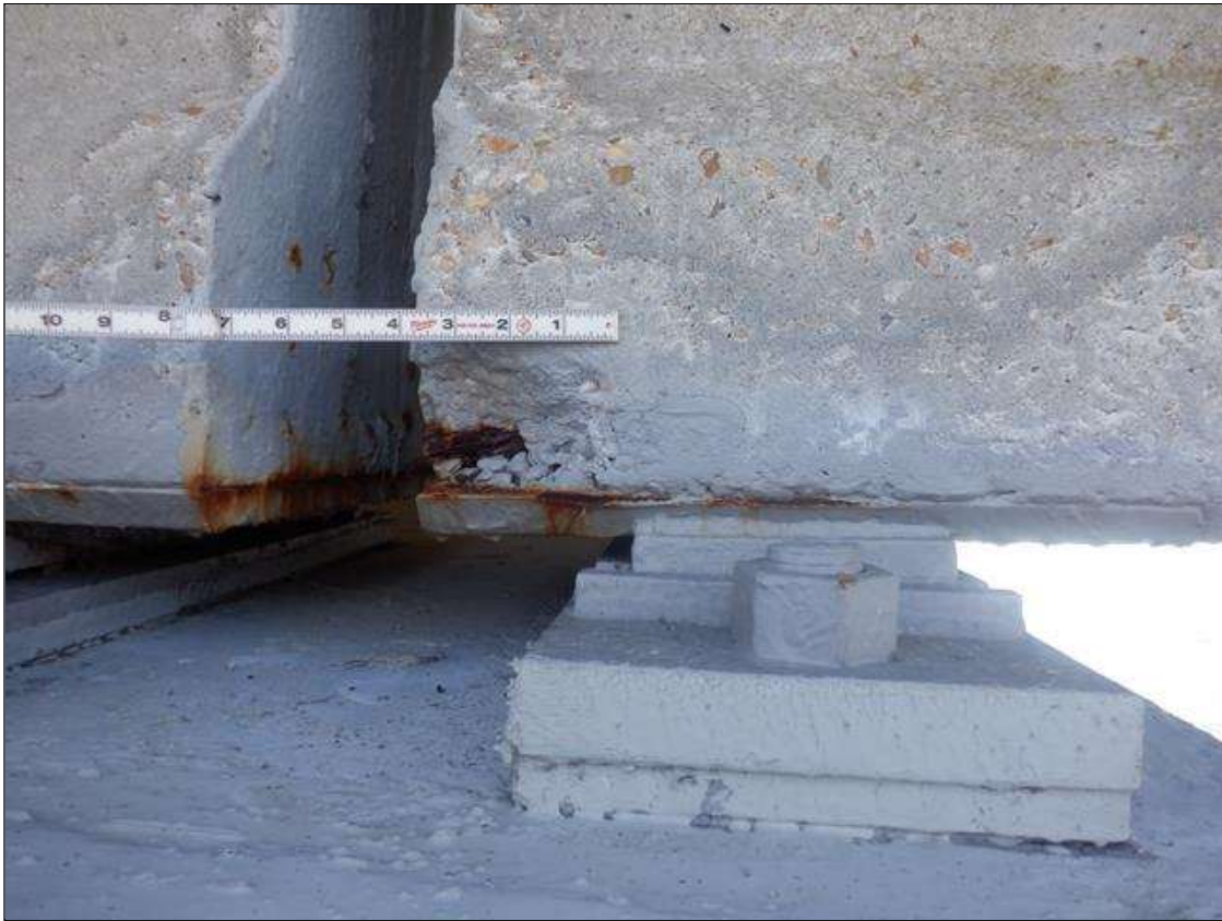
Span 192 Beam 1: (PAR) NORTH FACE BOTTOM FLANGE AT BEAM END, SPALL (3 INCHES DIAMETER X 2 INCHES DEEP) WITH ONE (1) EXPOSED STARND (25 PERCENT LOSS)
