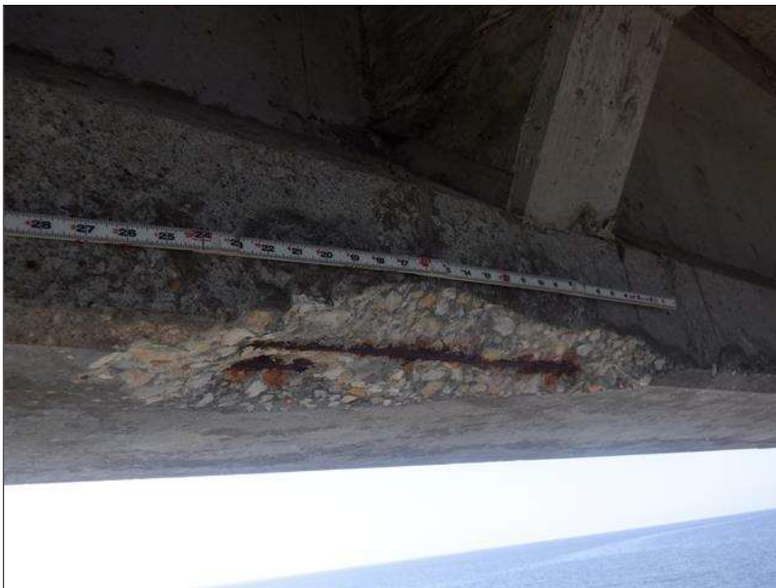
Span 184 Beam 4: (PAR) UNDERSIDE OF BOTTOM FLANGE AT 24 FEET FROM BENT 183, DELAMINATION/SPALL (2 FEET X 6 INCHES X 1 1/2 INCHES DEEP) WITH TWO (2) EXPOSED STRANDS (10 PERCENT LOSS)
