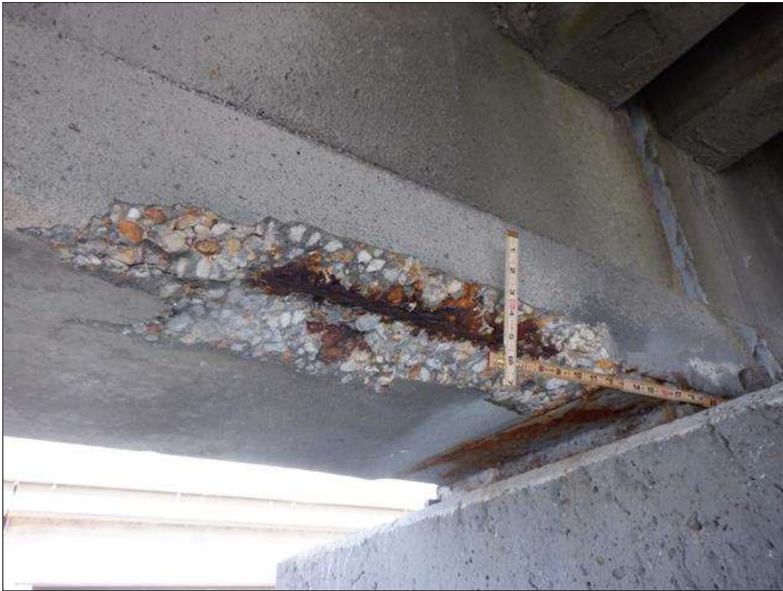
Span 111 Beam 1: (PAR) SOUTH FACE OF BOTTOM FLANGE AT BENT 111, DELAMINATION (20 INCHES X 3 INCHES) SOUTH FACE OF BOTTOM FLANGE AT BENT 111, SPALL (28 INCHES LONG X 4 INCHES HIGH X 8 INCHES ON BOTTOM X 1 1/2 INCHES DEEP) WITH (2) EXPOSED AND SEVERED STRANDS
