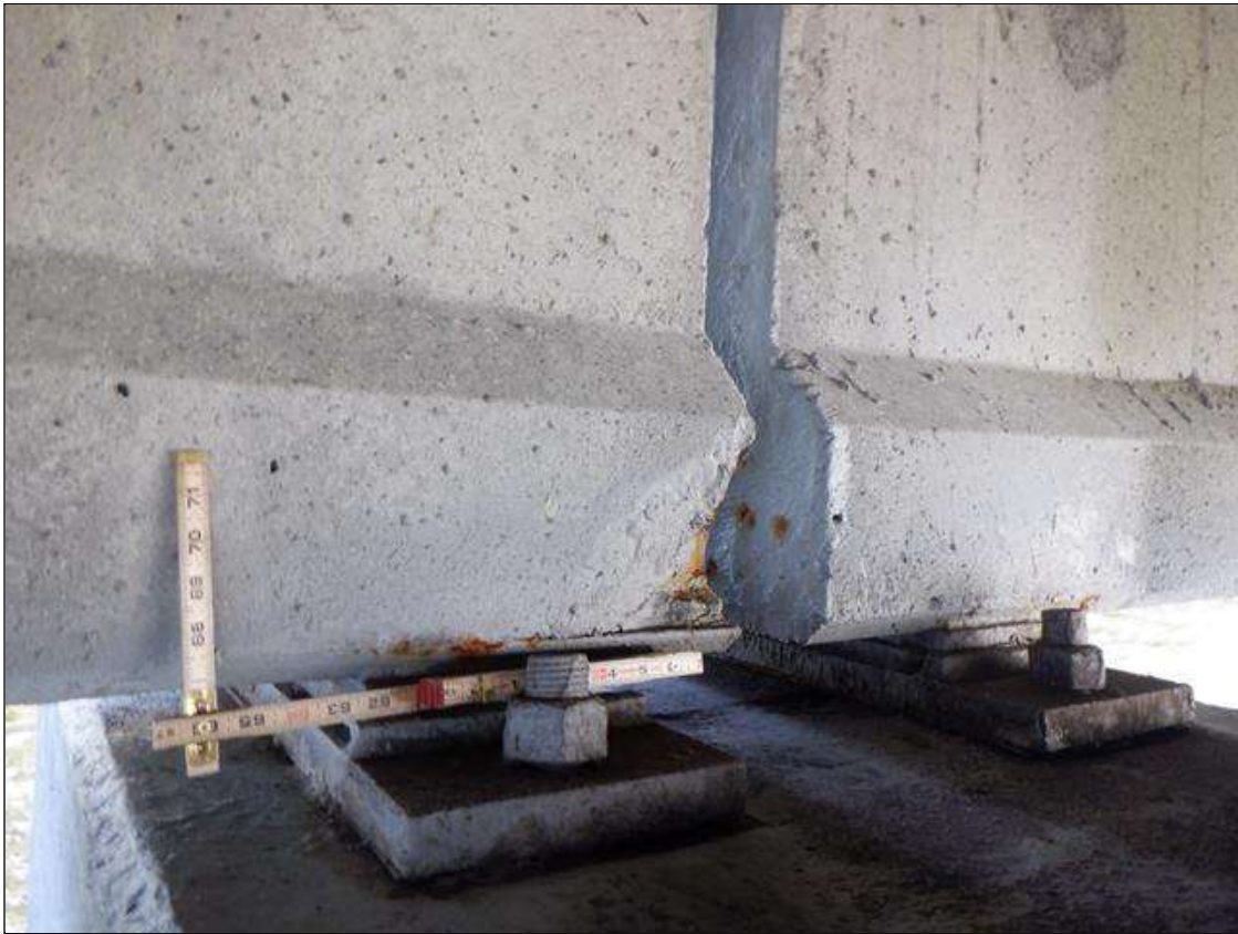
Span 116 Beam 1: (PAR) SOUTH FACE OF BOTTOM FLANGE, AT BENT 116, SPALL (7 INCHES X 7 INCHES X 3 INCHES) WITH EXPOSED STRANDS (5 PERCENT SECTION LOSS) ON STRAND
