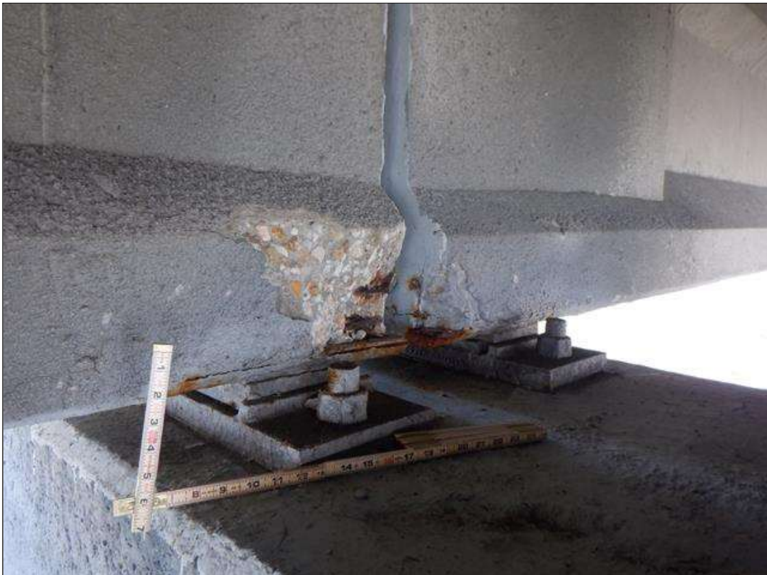
Span 109 Beam 1: (PAR) SOUTH FACE OF BOTTOM FLANGE AT BENT 109, SPALL (12 INCHES X 7 INCHES X 2.5 INCHES) WITH EXPOSED STRANDS (5 PERCENT SECTION LOSS) ON STRANDS
