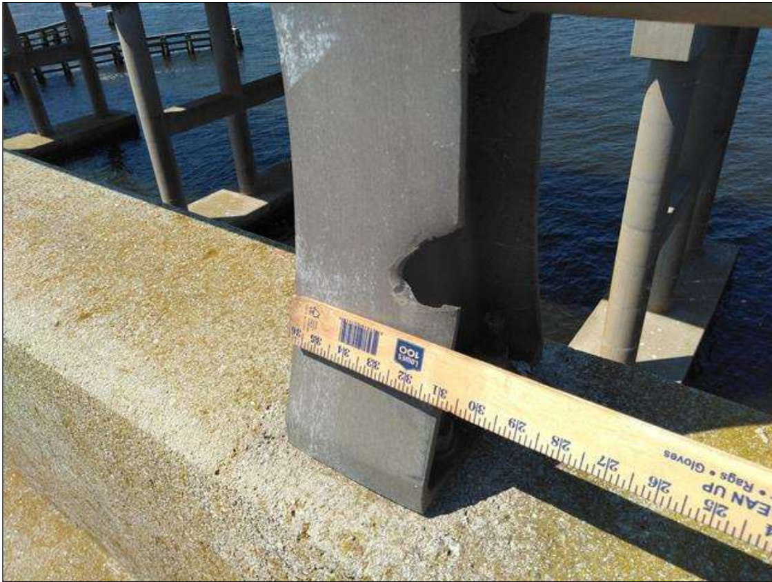
Span 183 Left Bridge Rail: RAILPOST 2, IMPACT DAMAGE (2 INCHES)
