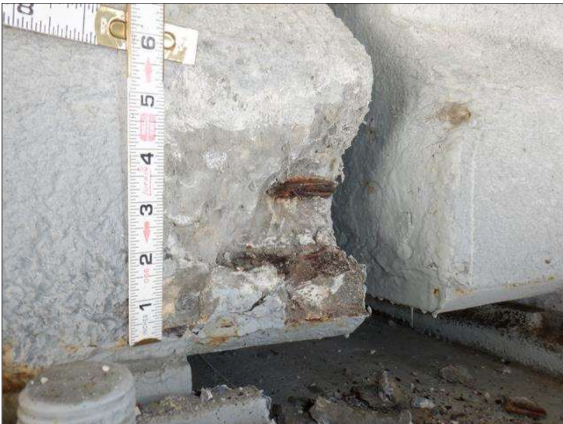
Span 21 Beam 3: (PAR) BOTTOM FLANGE SOUTH FACE AT BENT 21, SPALL (6 INCHES X 6 INCHES X UP TO 2 INCHES DEEP) WITH EXPOSED RUSTED STRANDS (20 PERCENT SECTION LOSS)
