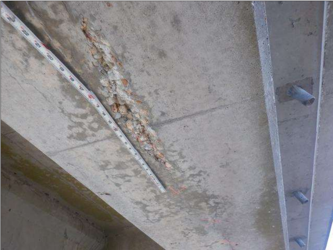
Span 175 Beam 1: UNDERSIDE OF BOTTOM FLANGE BEGINNING AT MIDSPAN, (2) LONGITUDINAL CRACKS (30 FEET X 0.01 INCHES) WITH ADJACENT SPALL (2 FEET X 1/2 INCH X 1/2 INCH DEEP)
