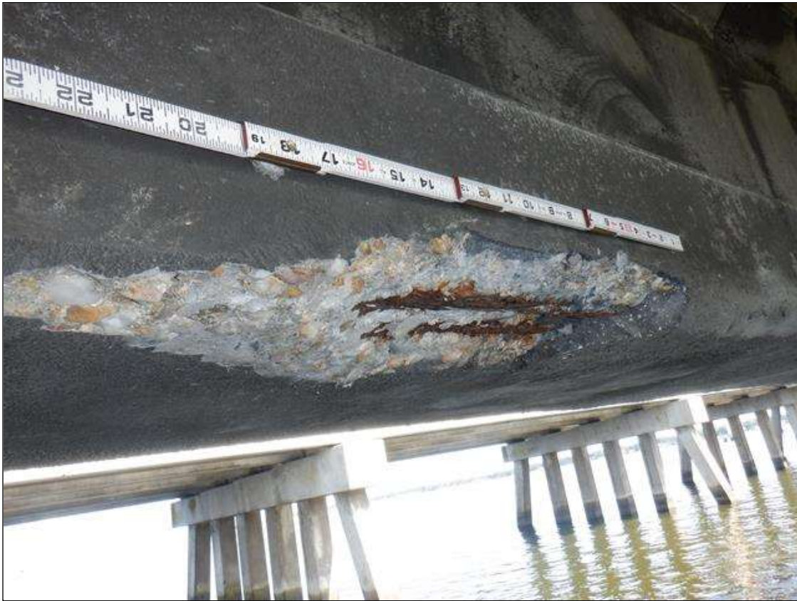
Span 160 Beam 1: (PAR) BOTH FACES OF BOTTOM FLANGE AT MIDSPAN, FAILED PATCH/SPALL (84 INCHES X 8 INCHES HIGH X UP TO 2 INCHES DEEP) WITH EXPOSED RUSTED STRANDS (30 PERCENT SECTION LOSS)
