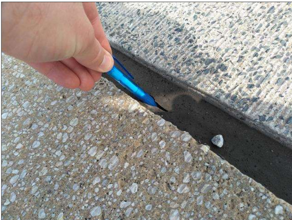
Span 154 Expansion Joint Bent 153: AT BENT 153, 3 CRACKS SCATTERED THROUGHOUT UP TO 2 INCH X FULL DEPTH
