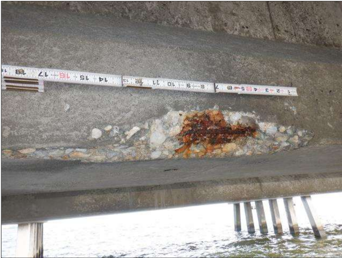
Span 51 Beam 2: (PAR) SOUTH FACE OF BOTTOM FLANGE, AT 10 FEET FROM BENT 50, SPALL (20 INCHES X 5 INCHES X 2 INCHES) WITH EXPOSED RUSTED STRAND (10 PERCENT SECTION LOSS)
