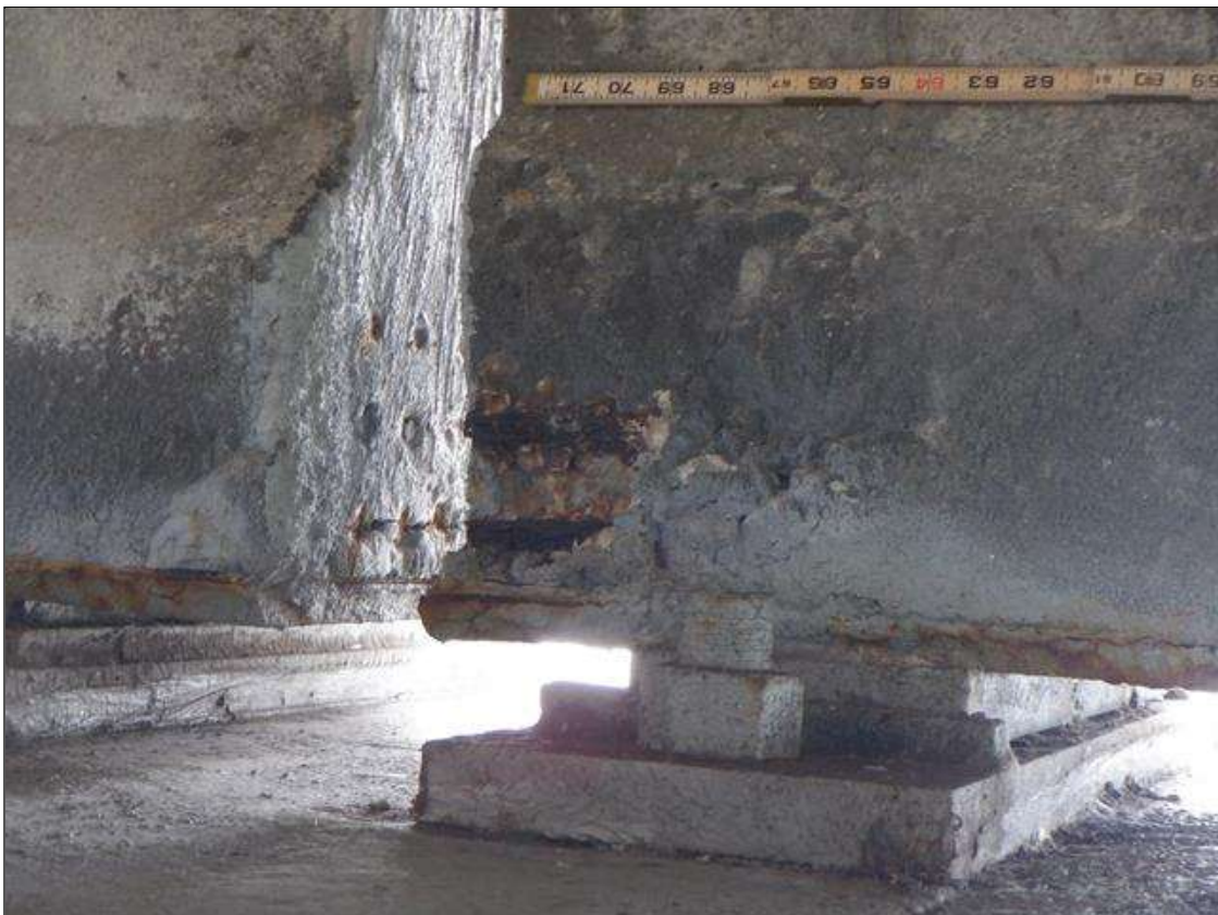
Span 102 Beam 4: (PAR) NORTH FACE OF BOTTOM FLANGE AT BENT 102, SPALL (10 INCHES LONG X 7 INCHES HIGH X 2 INCHES DEEP WITH (2) EXPOSED STRANDS (NO LOSS)
