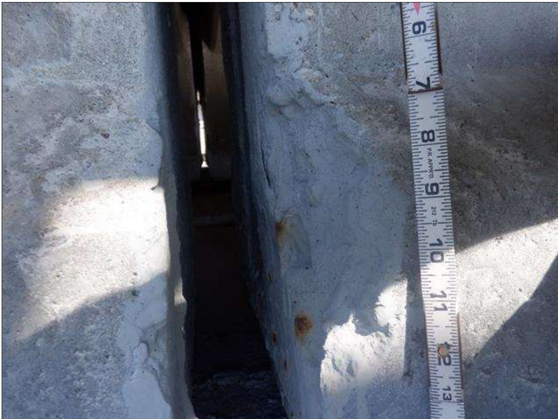
Span 98 Beam 4: BOTTOM FLANGE SOUTH FACE, AT BENT 97, SPALL (3 INCHES X 8 INCHES X 2 INCHES) WITH EXPOSED STRANDS (NO SECTION LOSS)
