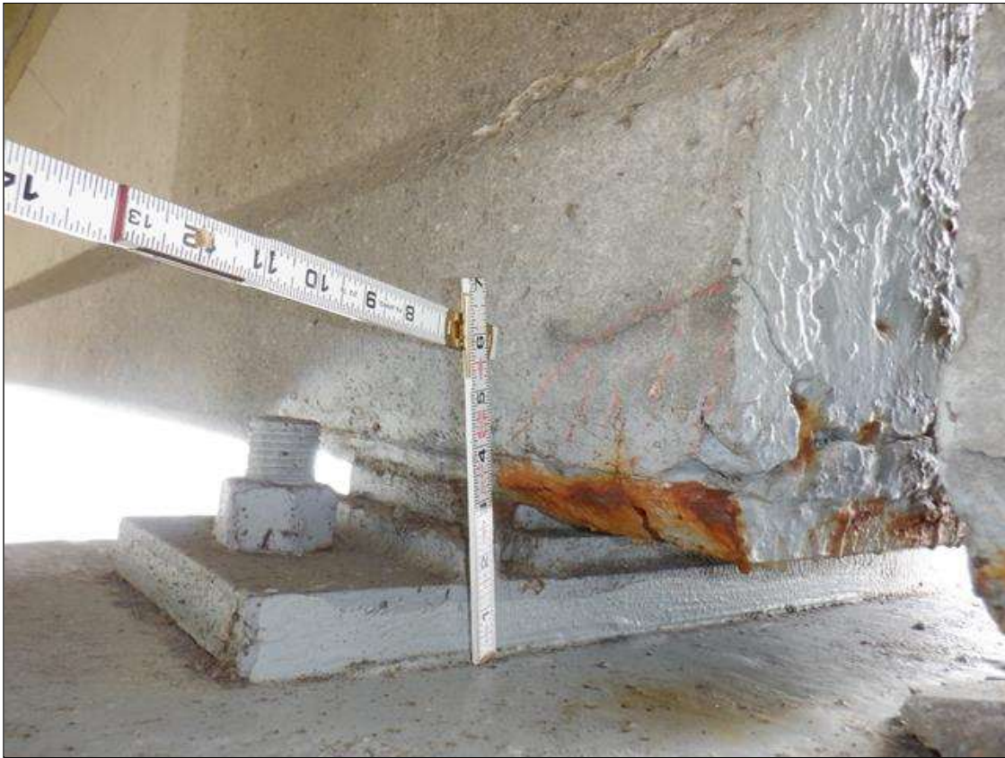
Span 22 Beam 4: NORTH FACE OF BOTTOM FLANGE, AT BENT 21, DELAMINATION (5 INCHES X 4 INCHES)
