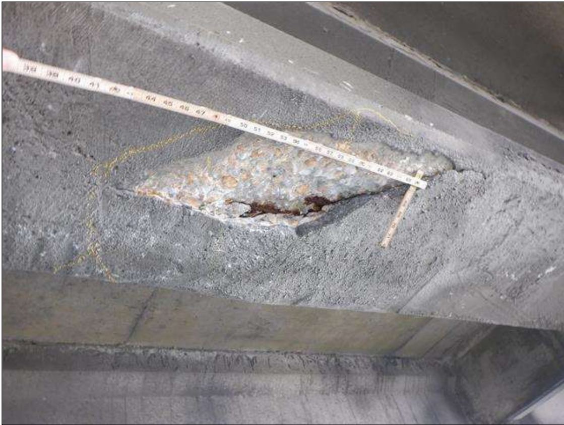
Span 138 Beam 2: (PAR) BOTTOM OF BOTTOM FLANGE AT 7 FEET FROM BENT 137, SPALL/DELAMINATION (37 INCHES LONG X FULL WIDTH X 2 INCHES DEEP) WITH (2) TWO EXPOSED STRANDS (10 PERCENT SECTION LOSS)
