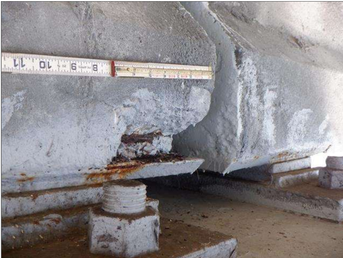
Span 221 Beam 3: SOUTH FACE OF BOTTOM FLANGE AT BENT 221, SPALL (4 INCHES X 8 INCHES X 2 INCHES) WITH EXPOSED RUSTED STRAND (30 PERCENT SECTION LOSS) ON STRAND
