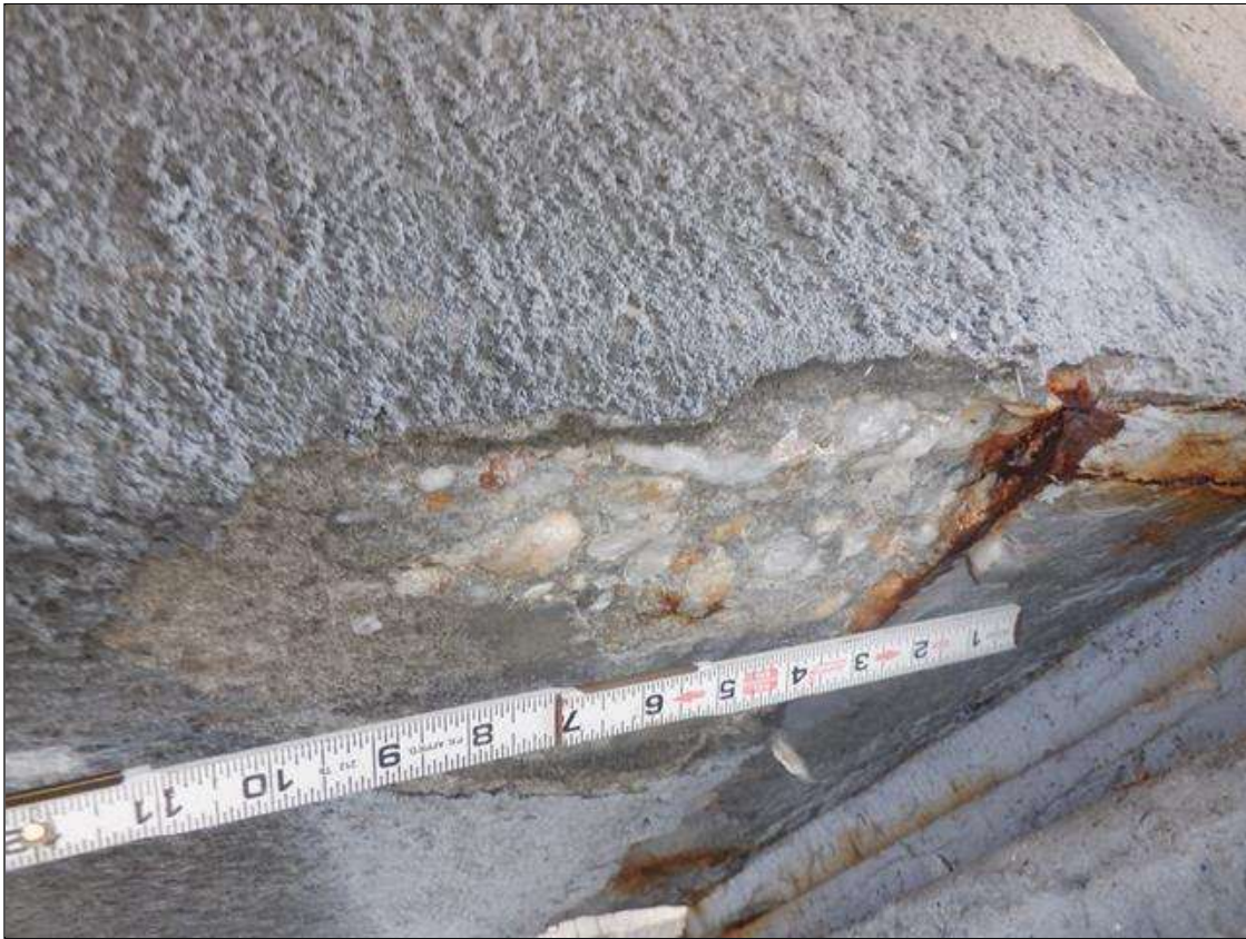
Span 98 Beam 3: UNDERSIDE OF BOTTOM FLANGE AT BENT 98, SPALL (6 INCHES X 3 INCHES X UP TO 1 INCH DEEP)
