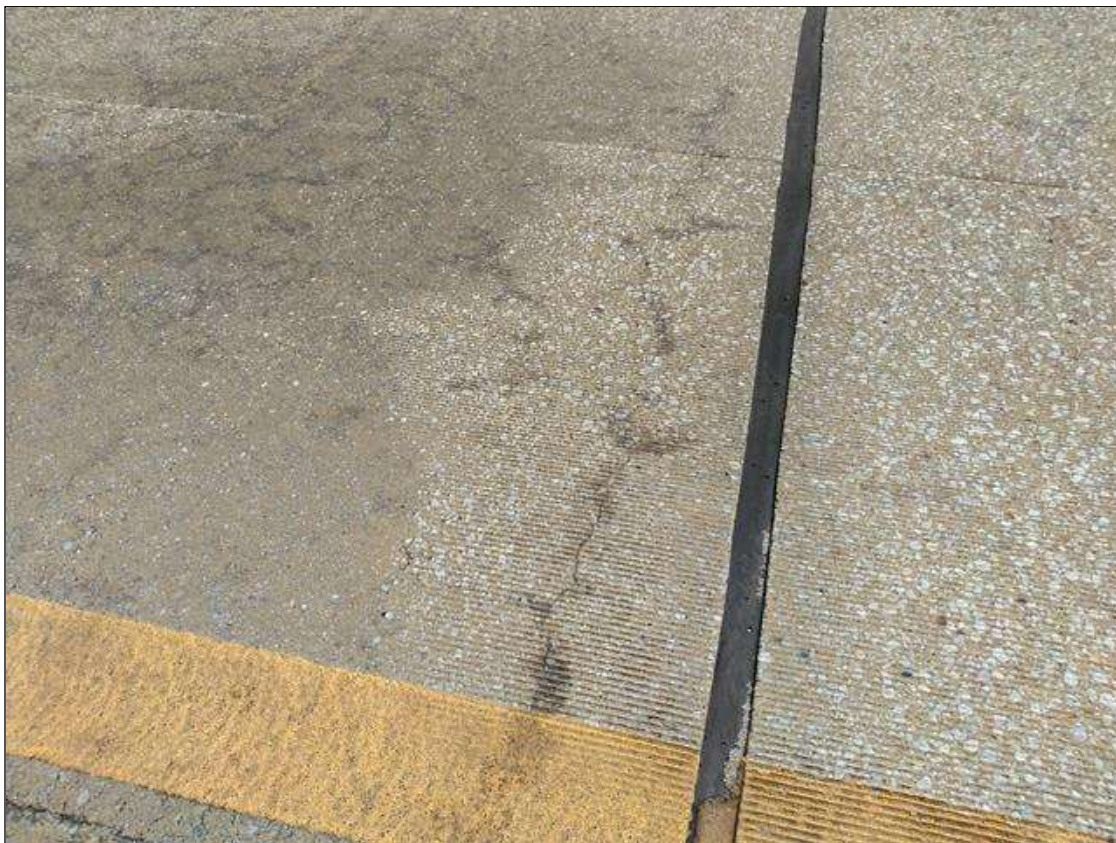
Span 62 Expansion Joint Bent 61: LEFT LANE NEAR CURB, DELAMINATION (4FEET X 6 INCHES)
