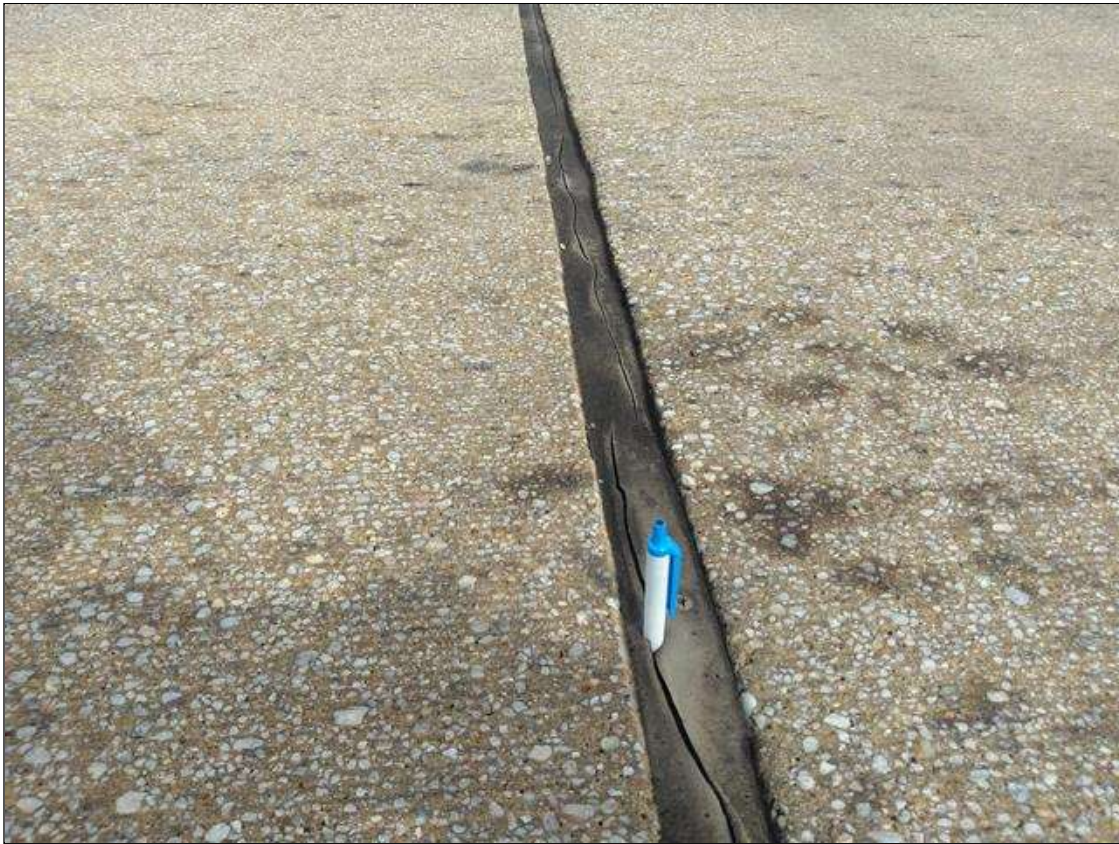
Span 237 Expansion Joint Bent 236: AT BENT 236, FULL DEPTH X FULL WIDTH CRACK
