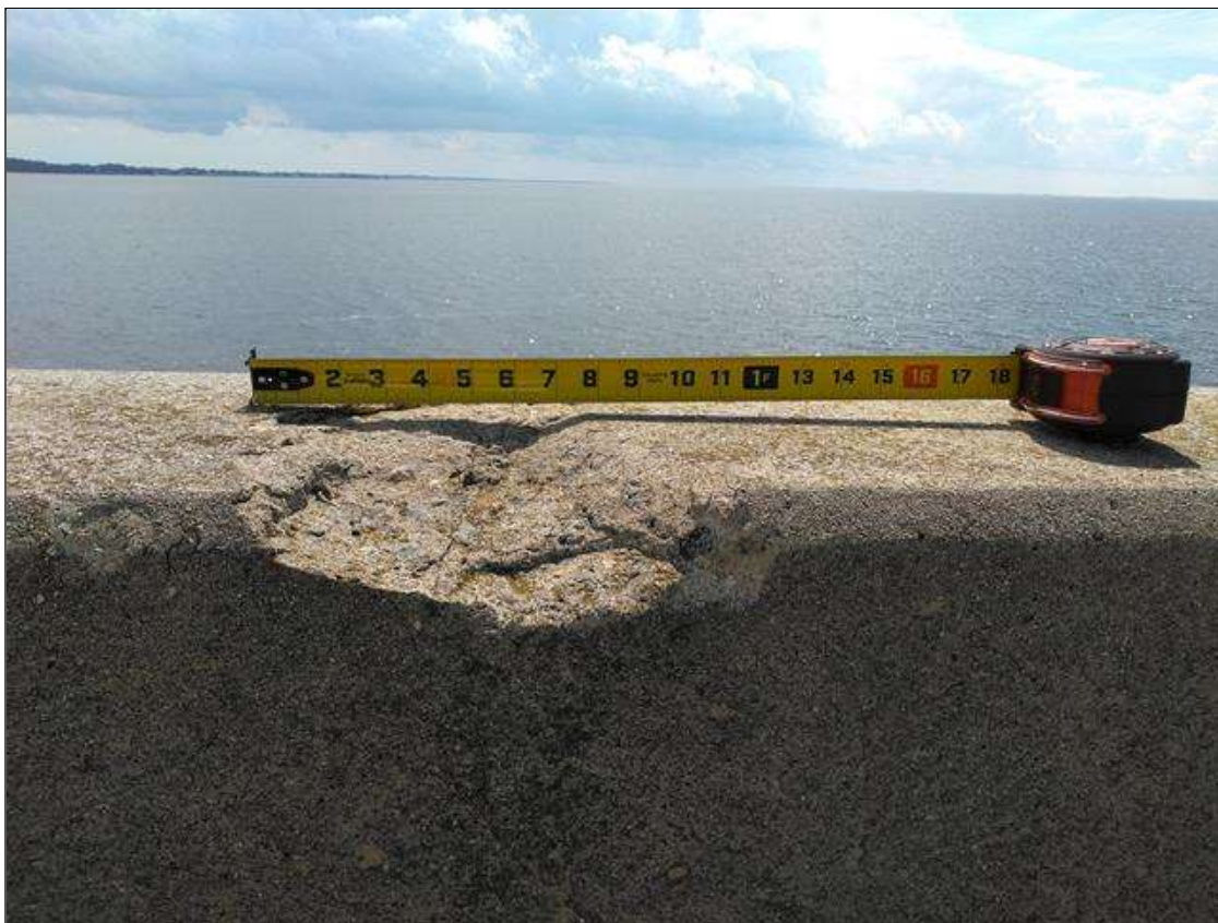
Span 173 Right Bridge Rail: TOP OF RAIL BETWEEN RAILPOSTS 2 AND 3, SPALL (16INCHES X 6INCHES X UP TO 1 INCHES). BETWEEN POSTS 3 AND 4, SPALL (9 INCH DIAMETER X 1.25 INCH DEEP)
