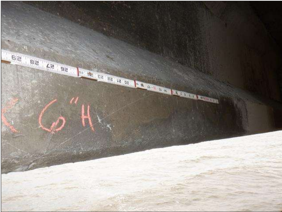
Span 71 Beam 4: NORTH FACE OF BOTTOM FLANGE AT 10 FEET FROM BENT 71, SOUND PATCH (36 INCHES X 6 INCHES)
