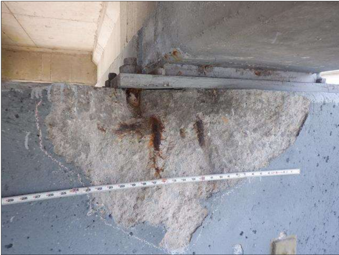
Bent 179 Cap 1: (PAR) TOP OF EAST FACE BELOW GIRDER 1, SPALL (30 INCHES X 16 INCHES X UP TO 8 INCHES DEEP) WITH TWO (2) EXPOSED STIRRUPS AND ONE (1) EXPOSED ANCHOR BOLT, EXTENDING BELOW BEARING (UP TO 10 PERCENT) WITH UNDERMINING OF MASONRY PLATE (7 INCHES X 3 INCHES AVERAGE)
