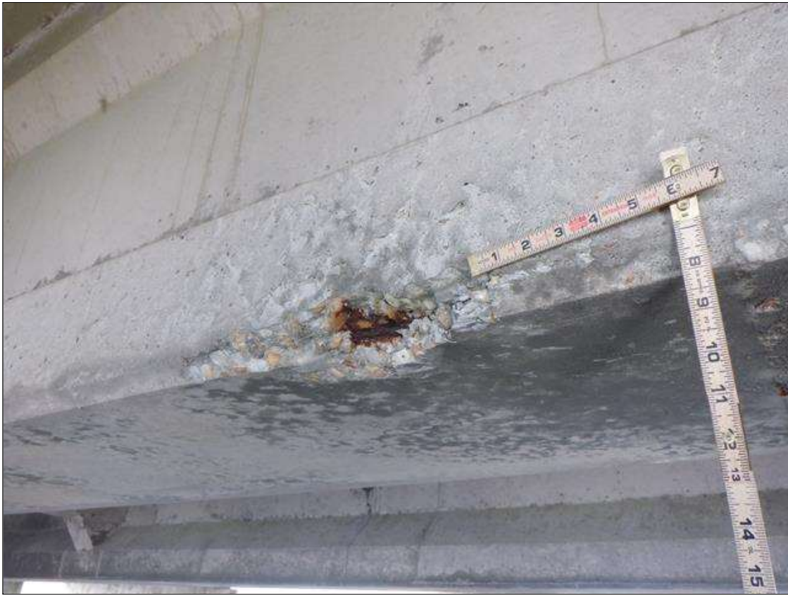
Span 121 Beam 2: (PAR) BOTTOM OF BOTTOM FLANGE AT MIDSPAN, SPALL/DELAMINATION (20 INCHES LONG X 3 INCHES HIGH X 5 INCHES WIDE X 1.5 INCHES DEEP) WITH (1) EXPOSED RUSTED STRAND (10 PERCENT SECTION LOSS)
