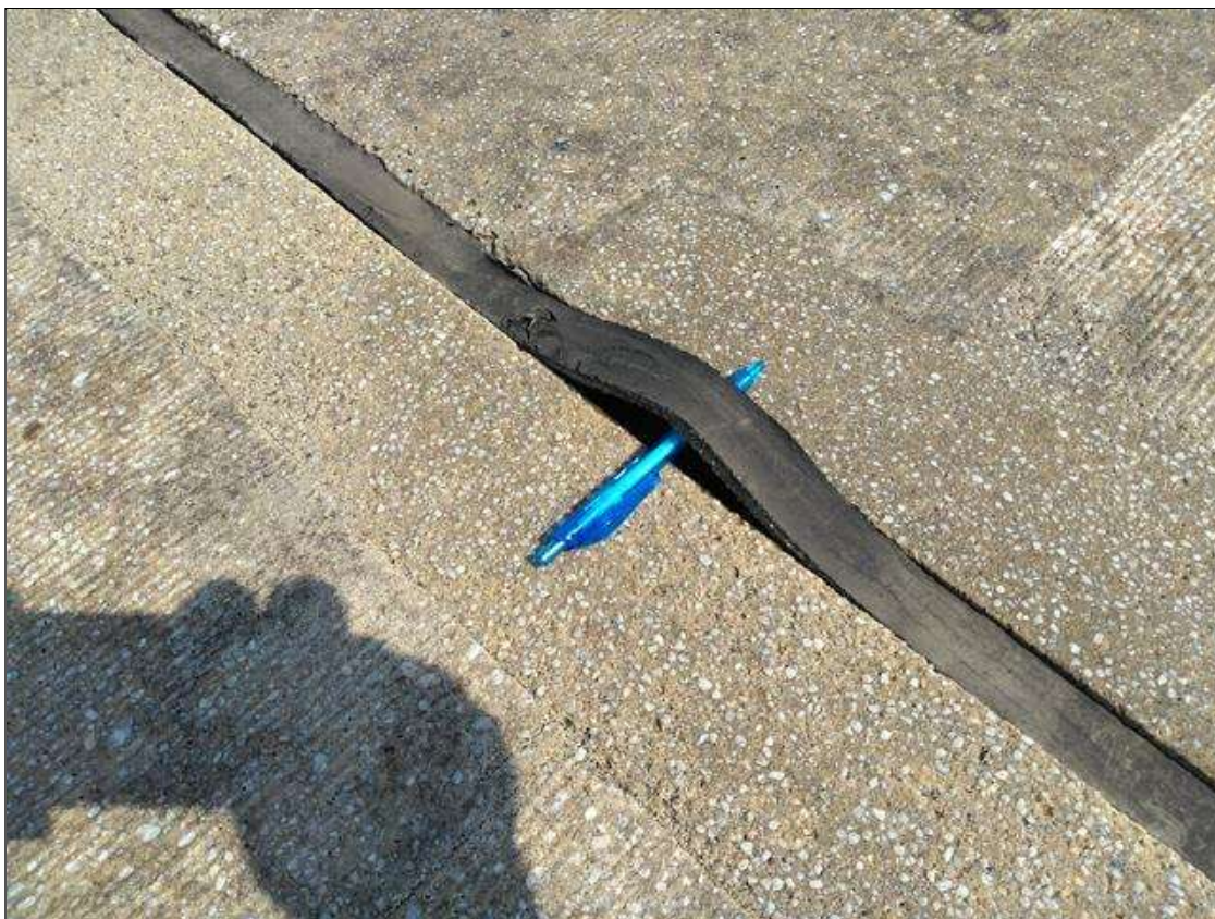
Span 145 Expansion Joint Bent 144: LEFT LANE NEAR CENTERLINE OF ROADWAY, PATCHED AREA (4FEET X 4 INCHES), NO JOINT ADHESION AT PATCH
