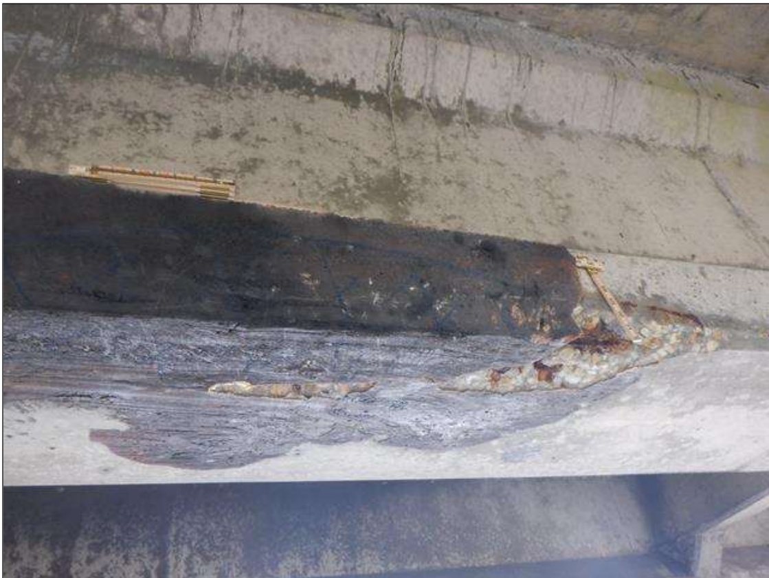
Span 152 Beam 2: (PAR) NORTH FACE OF BOTTOM FLANGE AT 12 FEET FROM BENT 152, SPALL (18 INCHES X 8 INCHES X 2 INCHES) WITH EXPOSED RUSTED STRANDS (75 PERCENT SECTION LOSS)
