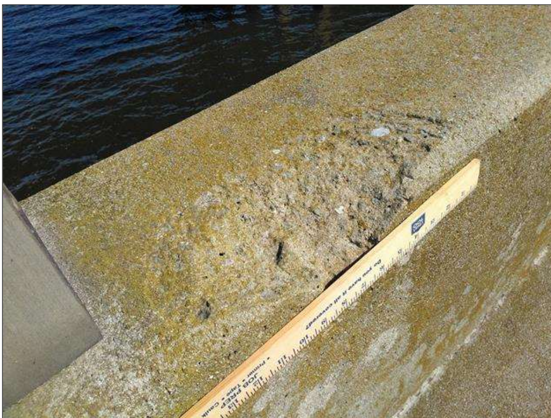
Span 21 Left Bridge Rail: RAIL AT RAILPOST 4, SPALL (12INCHES X 6INCHES X 1 INCHES)
