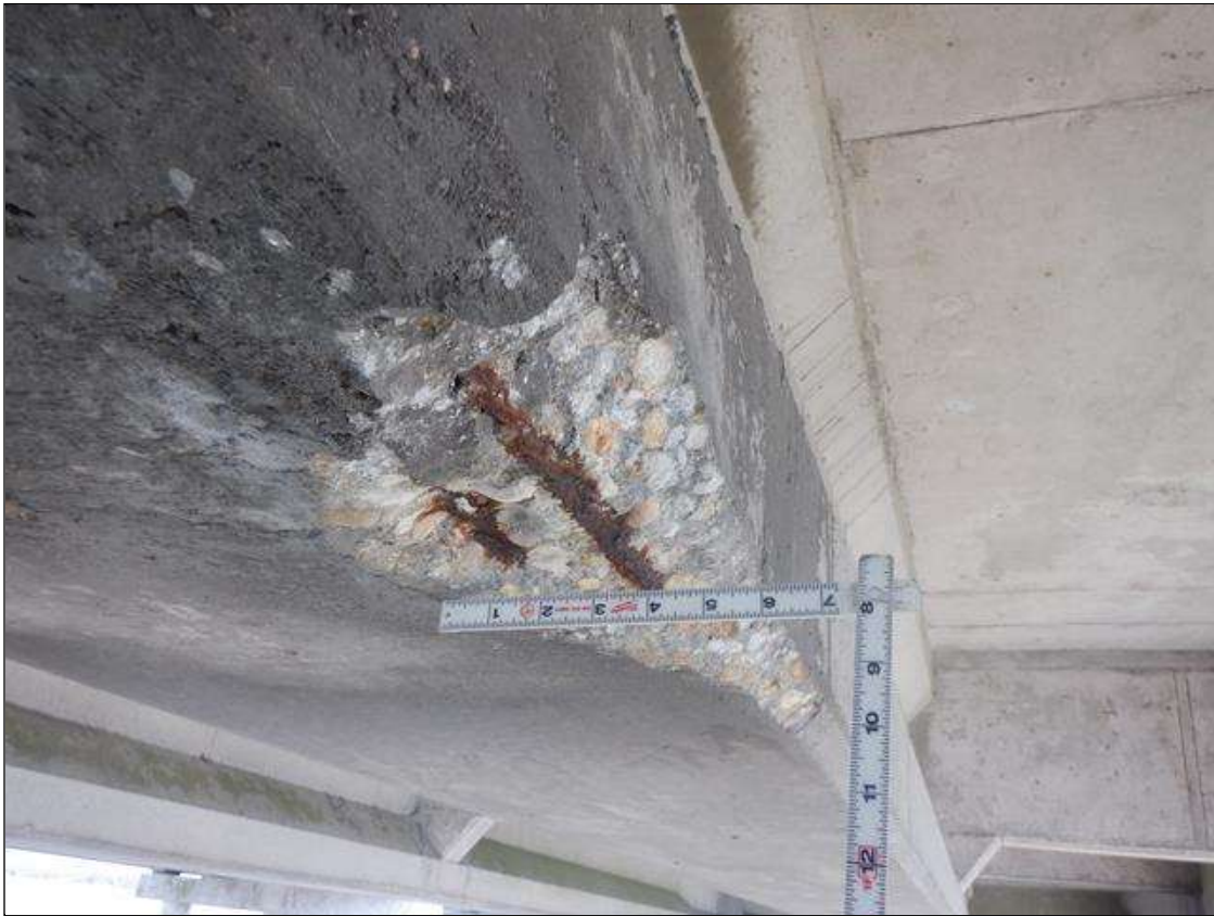
Span 180 Beam 2: (PAR) BOTTOM FLANGE SOUTH FACE AT 22 FEET FROM BENT 179, SPALL (12 INCHES X 6 INCHES X 1.5 INCHES DEEP) WITH TWO (2) EXPOSED RUSTED STRANDS (10 PERCENT SECTION LOSS)
