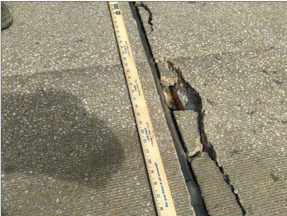
Span 31 Expansion Joint Bent 30: (PAR) AT BENT 30, RIGHT LANE SPALL 4 FEET WIDE X 6 INCH LONG X 5 INCHES DEEP WITH EXPOSED REBAR
