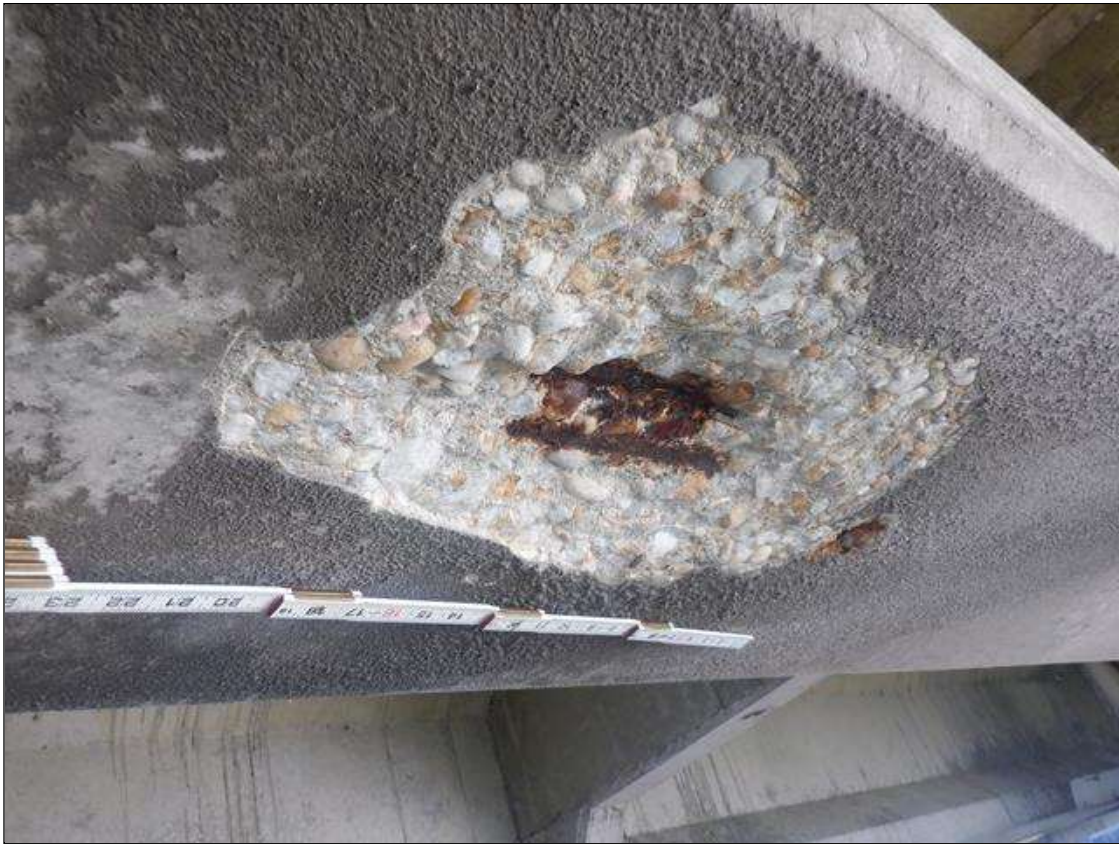
Span 97 Beam 2: (PAR) BOTTOM FLANGE AT 24 FEET FROM BENT 97, SPALL (19 INCHES X 12 INCHES X 1 INCHES) WITH EXPOSED STRANDS (10 PERCENT SECTION LOSS) ON STRAND
