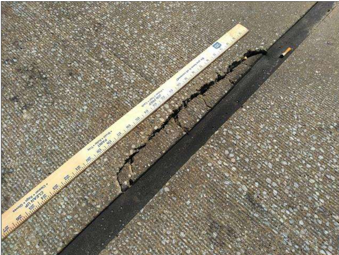
Span 53 Expansion Joint Bent 52: (PAR) AT BENT 52, RIGHT LANE 20 INCH LONG X 2 INCH WIDE SPALL AND DELAMINATION
