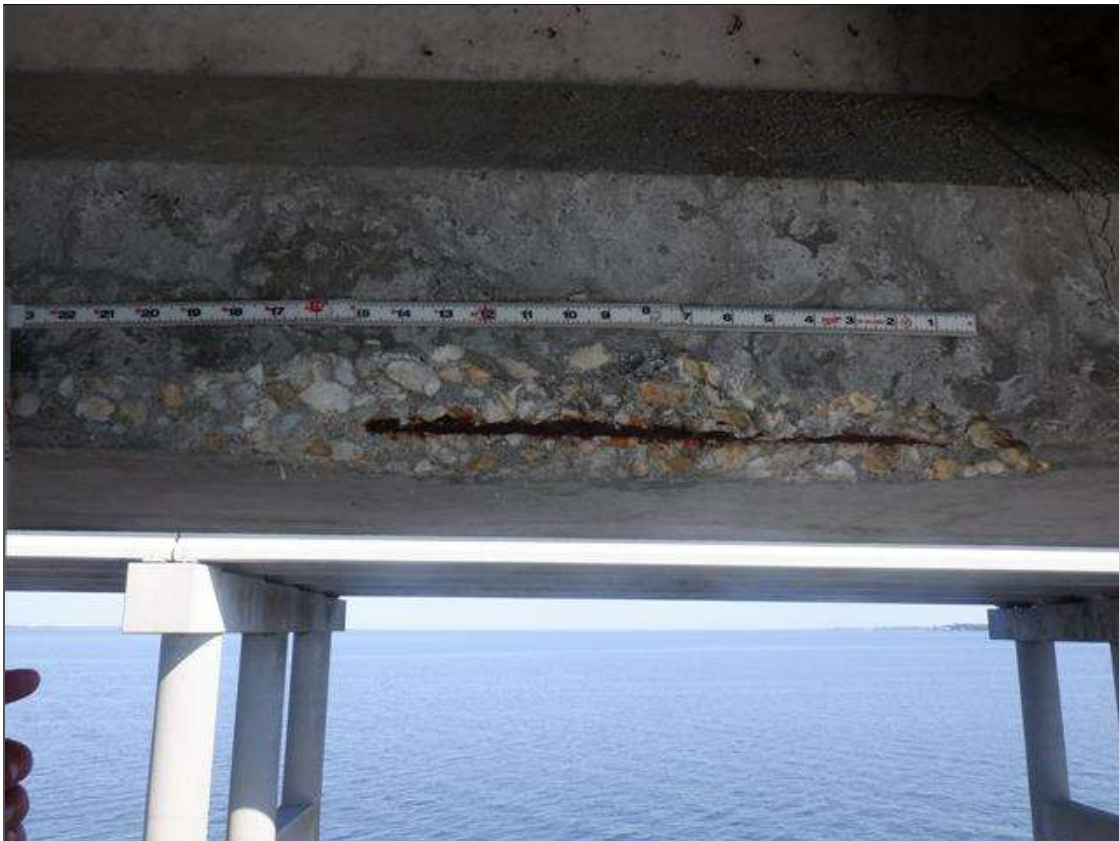
Span 183 Beam 1: (PAR) BOTTOM FLANGE SOUTH FACE 24 FEET EAST OF BENT 182, SPALL (2 FEET X 4 INCHES X 1 1/2 INCHES DEEP) WITH ONE (1) EXPOSED STRAND (10 PERCENT LOSS)
