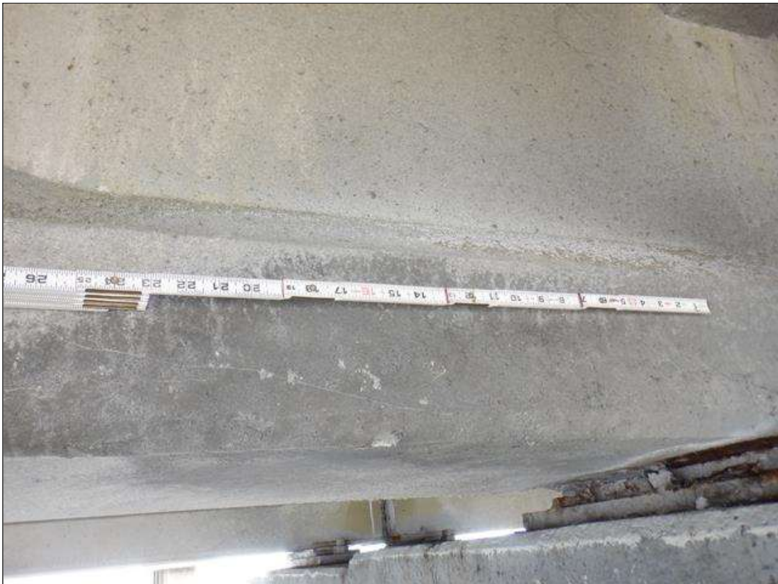
Span 66 Beam 2: SOUTH FACE OF BOTTOM FLANGE AT BENT 66, SOUND PATCH (2 FEET X 4 INCHES)
