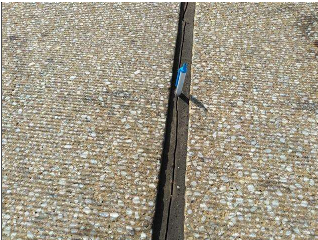
Span 224 Expansion Joint Bent 223: AT BENT 223 FULL DEPTH X FULL WIDTH CRACK
