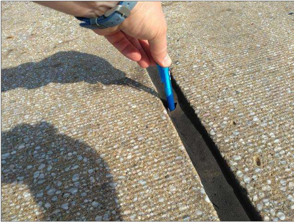
Span 118 Expansion Joint Bent 117: BENT 117, 1 INCH LONG FULL DEPTH CRACK LEFT LANE
