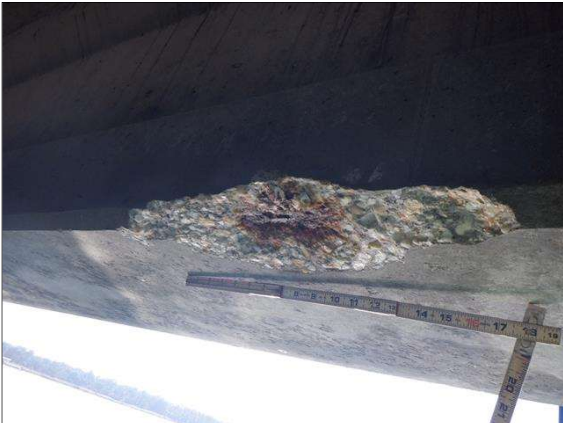
Span 217 Beam 4: (PAR) NORTH FACE OF BOTTOM FLANGE, AT 5 FEET FROM BENT 216, SPALL (18 INCHES X 4 INCHES X 2 INCHES) WITH EXPOSED STRANDS (10 PERCENT SECTION LOSS) ON STRAND
