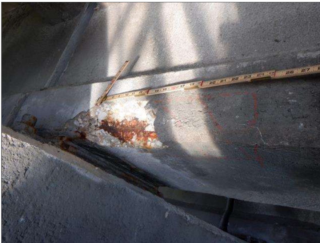
Span 104 Beam 3: (PAR) SOUTH FACE OF BOTTOM FLANGE AT BENT 103, DELAMINATION/SPALL (24 INCHES LONG X 4 INCHES HIGH X 4 INCHES ON BOTTOM FACE X 2 INCHES DEEP) WITH (1) EXPOSED STRAND (NO LOSS)
