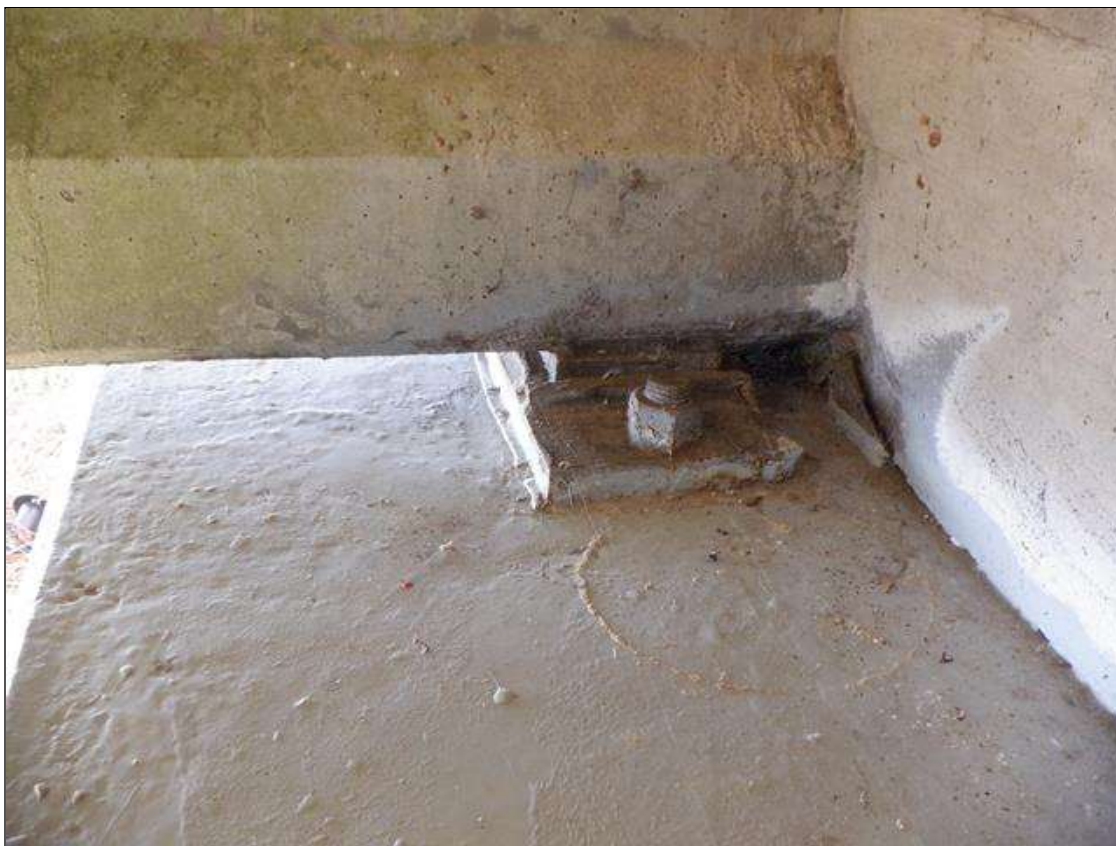
TYPICAL END BEARING
