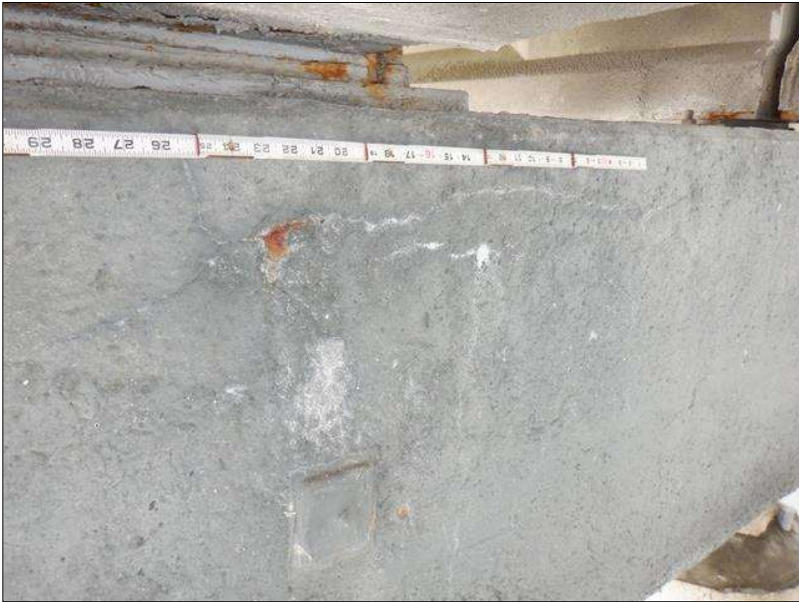
Bent 17 Cap 1: ALL FACES, SCATTERED PATCHED AREAS WITH MAP CRACKING (UP TO 1/32 INCHES), SOME WITH EFFLORESCENCE AND RUST STAIN
