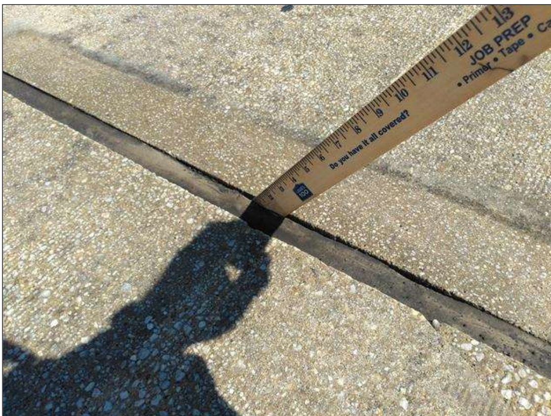
Span 37 Expansion Joint Bent 36: AT BENT 36, LEFT LANE PARTIAL DEPTH ADHESION LOSS 2 FEET LONG
