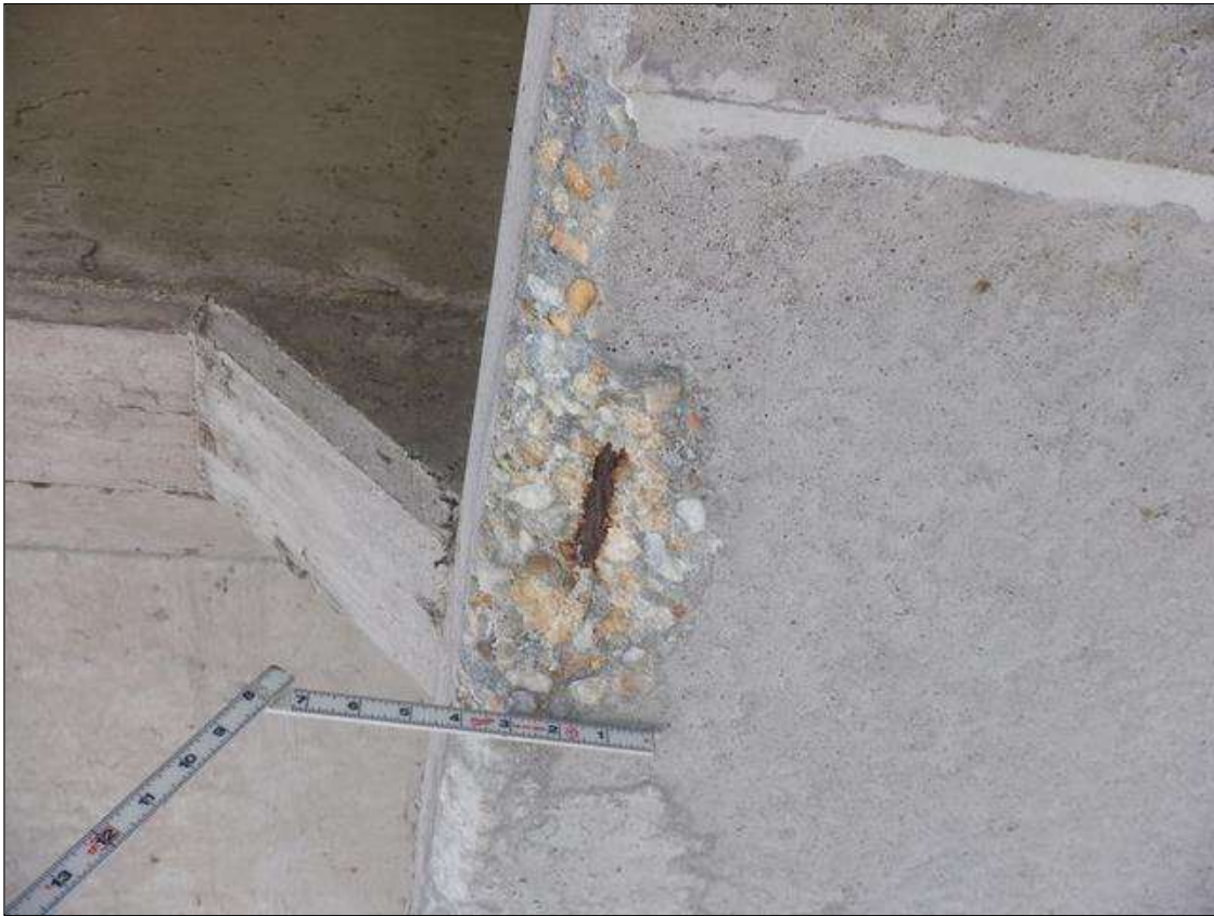
Span 177 Beam 3: SOUTH FACE OF BOTTOM FLANGE AT 23 FEET FROM BENT 177, SPALL (1 FOOT X 3 INCHES X 1 INCH DEEP) WITH ONE (1) EXPOSED RUSTED STRAND (NO SECTION LOSS)
