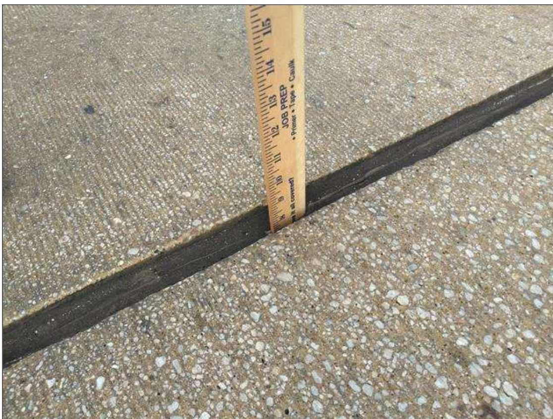
Span 105 Expansion Joint Bent 104: THROUGHOUT BOTH LANES, SEAL DAMAGED AND TORN
