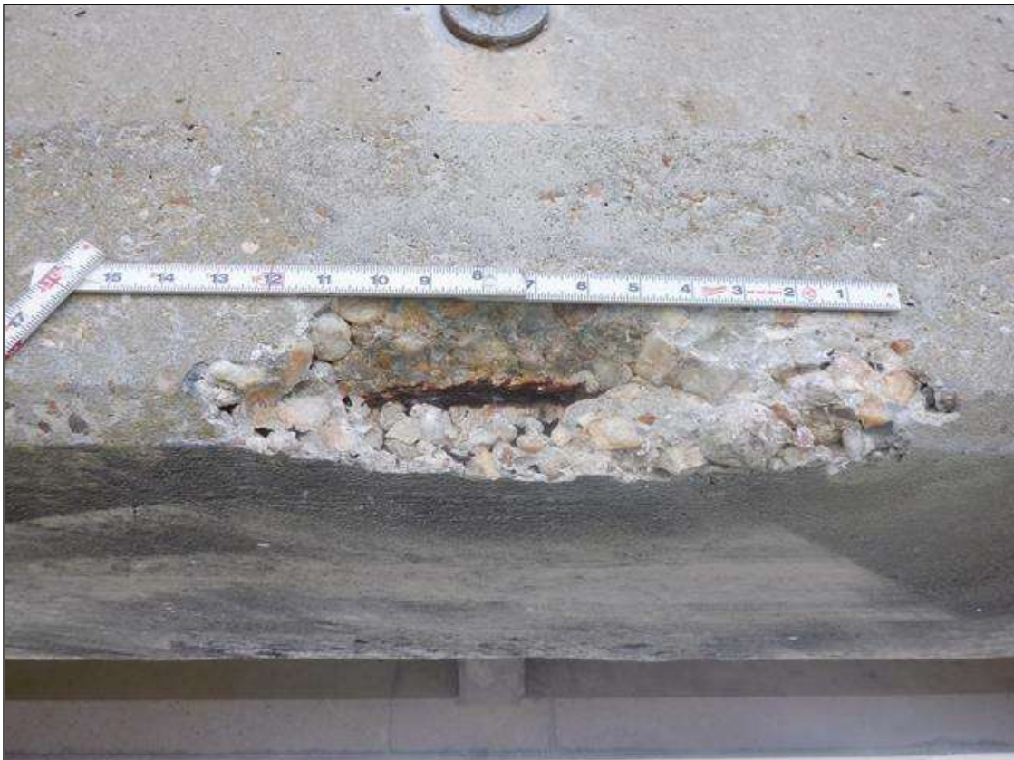
Span 193 Beam 1: (PAR) NORTH FACE BOTTOM FLANGE AT MIDSPAN, SPALL (1 FOOT X 2 INCHES X 2 INCHES DEEP) WITH ONE (1) EXPOSED STARND (25 PERCENT LOSS)
