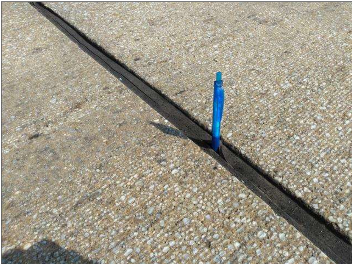
Span 129 Expansion Joint Bent 128: AT BENT 128, FULL DEPTH AND WIDTH CRACK
