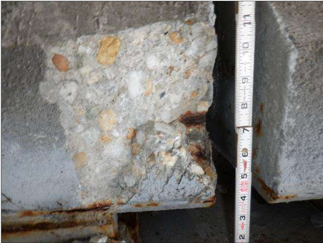
Span 85 Beam 2: SOUTH FACE OF BOTTOM FLANGE, BENT 85, SPALL (7 INCHES X 7 INCHES X 2 INCHES) WITH EXPOSED RUSTED STRANDS (NO SECTION LOSS)
