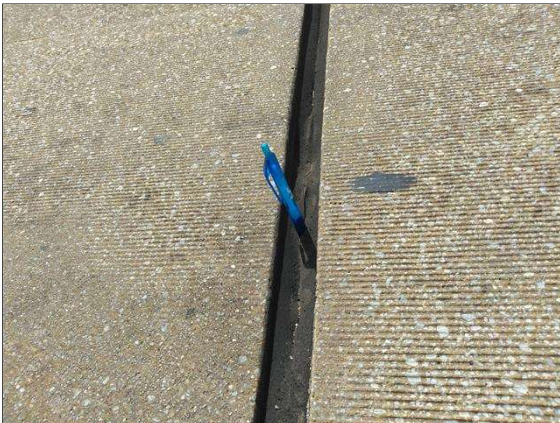
Span 136 Expansion Joint Bent 135: AT BENT 135, PARTIAL DEPTH CRACK IN LEFT LANE 1 FOOT LONG
