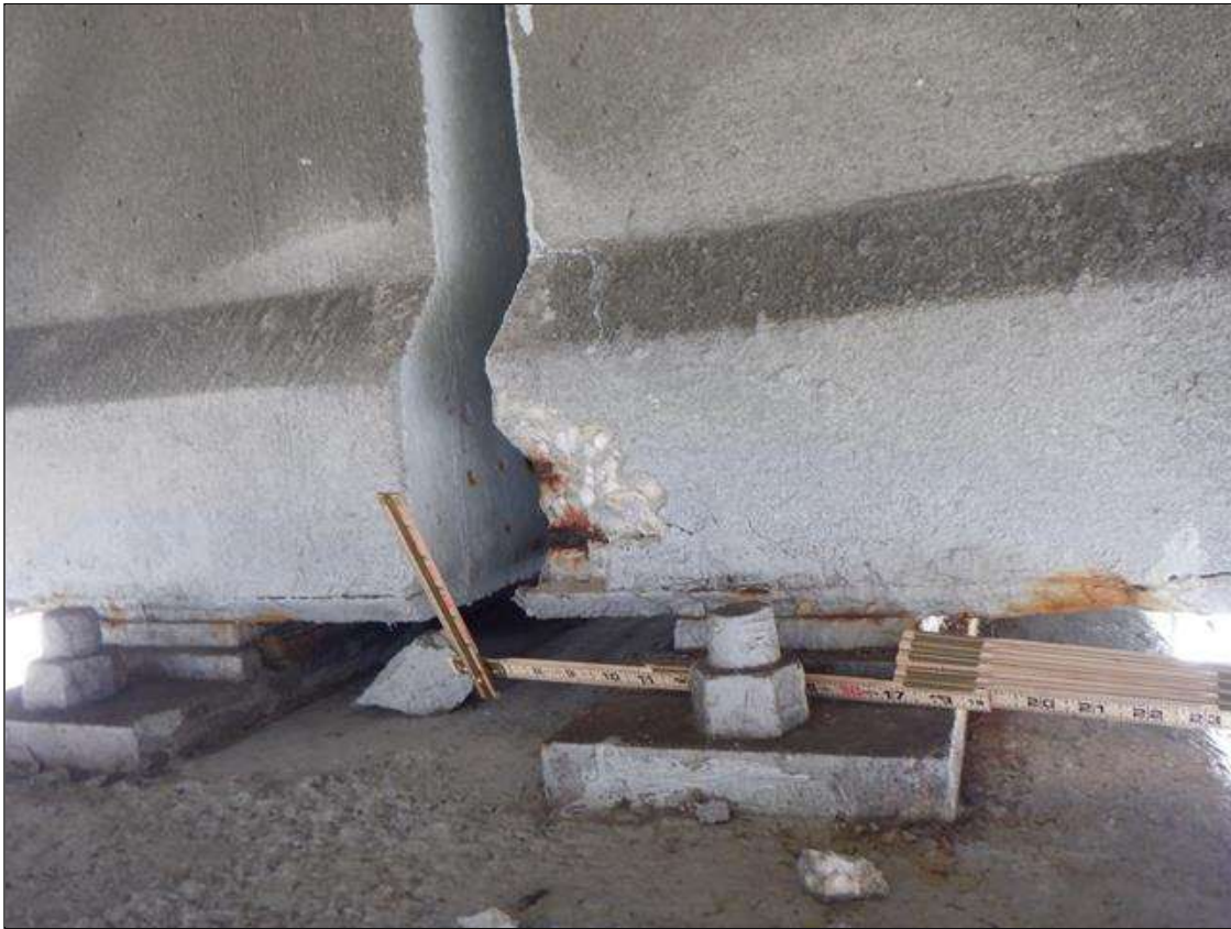
Span 123 Beam 2: (PAR) NORTH FACE OF BOTTOM FLANGE AT BENT 123, SPALL (5INCHES X 6INCHES X 2 INCHES) WITH (2) TWO EXPOSED STRANDS (5 PERCENT SECTION LOSS) ON STRAND
