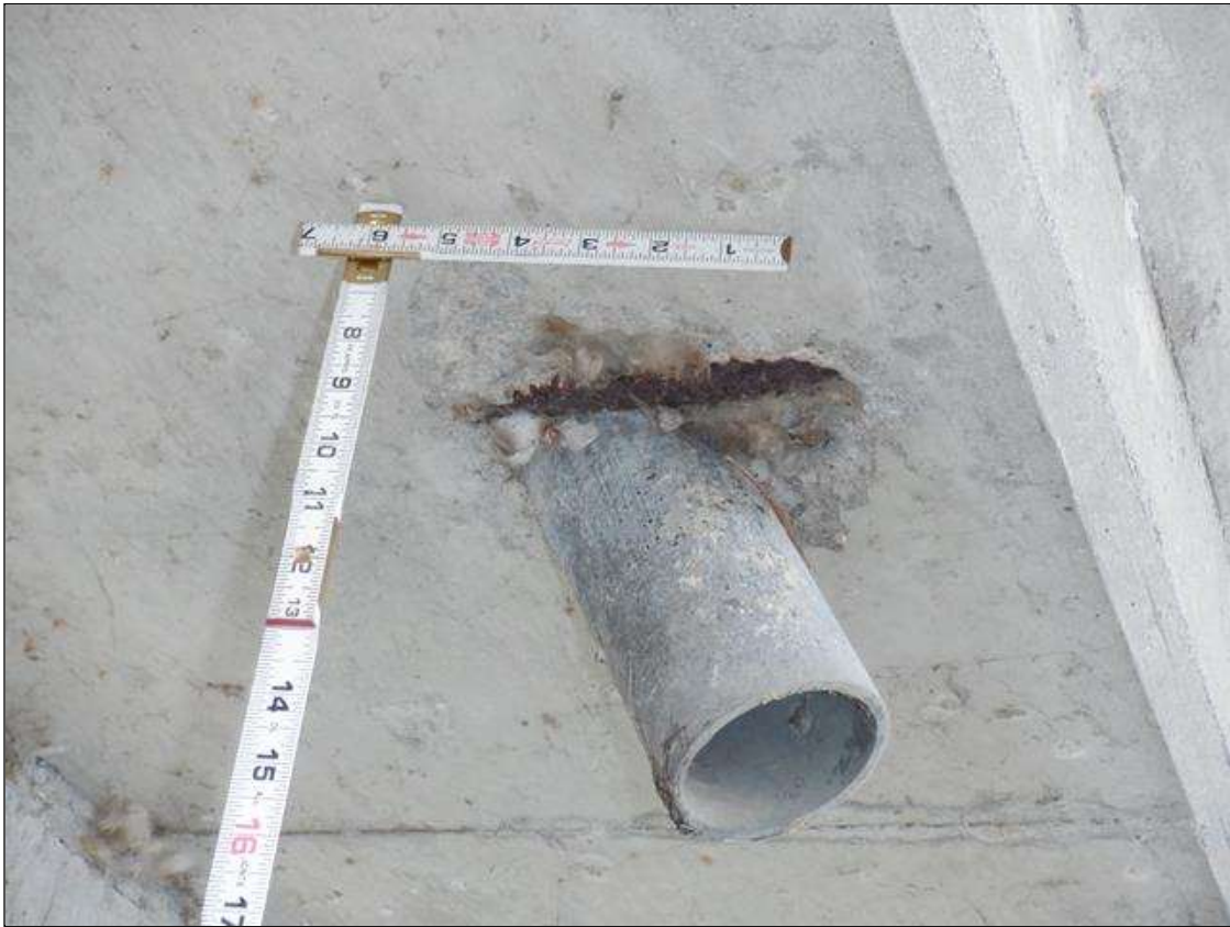
Span 16 Deck: UNDERSIDE OF RIGHT OVERHANG AT DRAIN DOWNSPOUT NEAR MIDSPAN, SPALL (6 INCH DIAMETER X 1/2 INCH DEEP) WITH EXPOSED RUSTED REINFORCING (NO SECTION LOSS)
