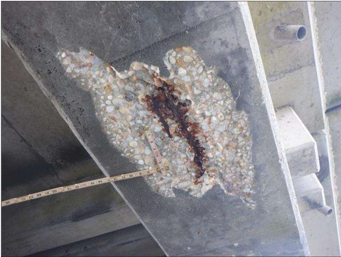
Span 104 Beam 1: (PAR) UNDERSIDE OF BOTTOM FLANGE 4 FEET FROM BENT 103, SPALL (66 INCHES X 14 INCHES X 1.5 INCHES) WITH EXPOSED STRANDS AND (1) BROKEN STRAND
