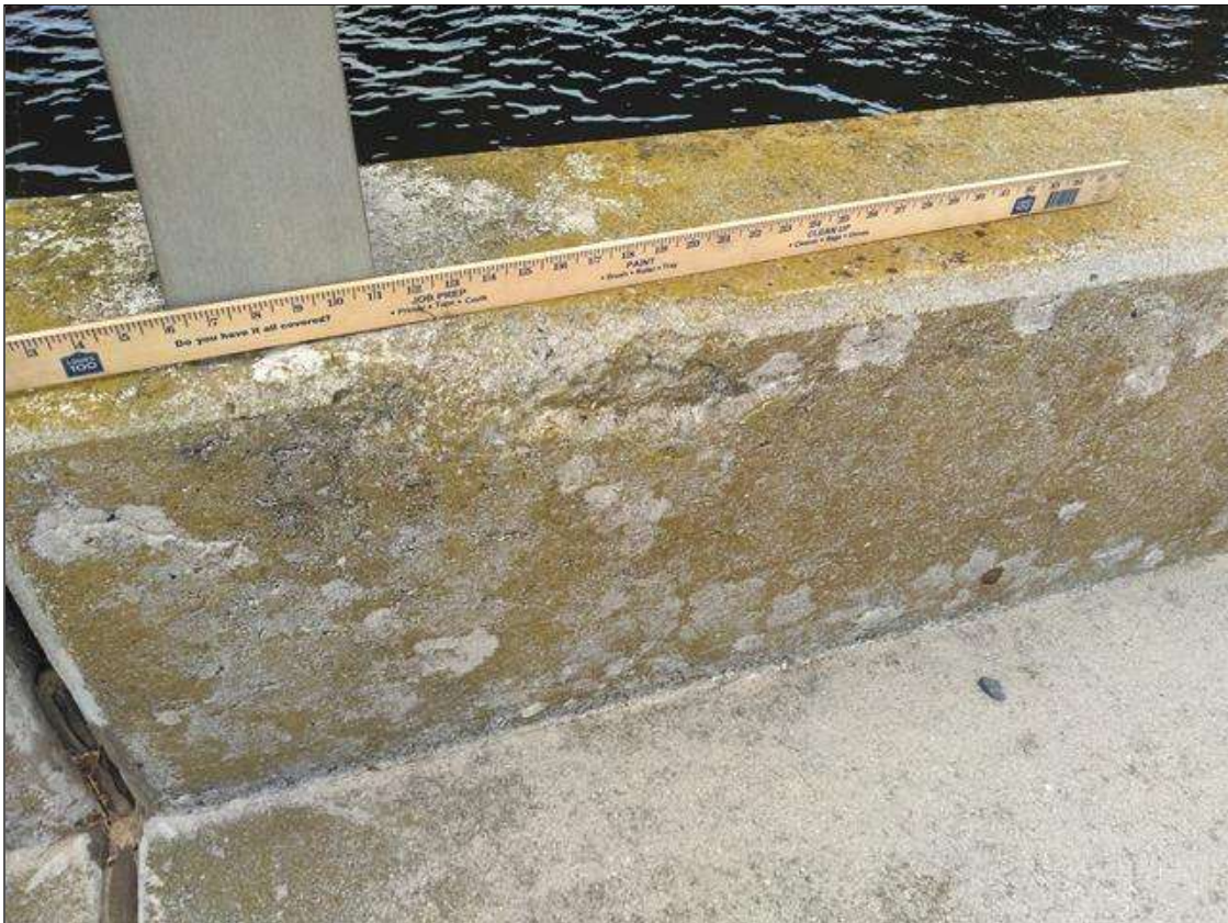
Span 79 Left Bridge Rail: AT RAILPOST 1, SPALL (UP TO 2FEET X 5INCHES X 1/2 INCHES)
