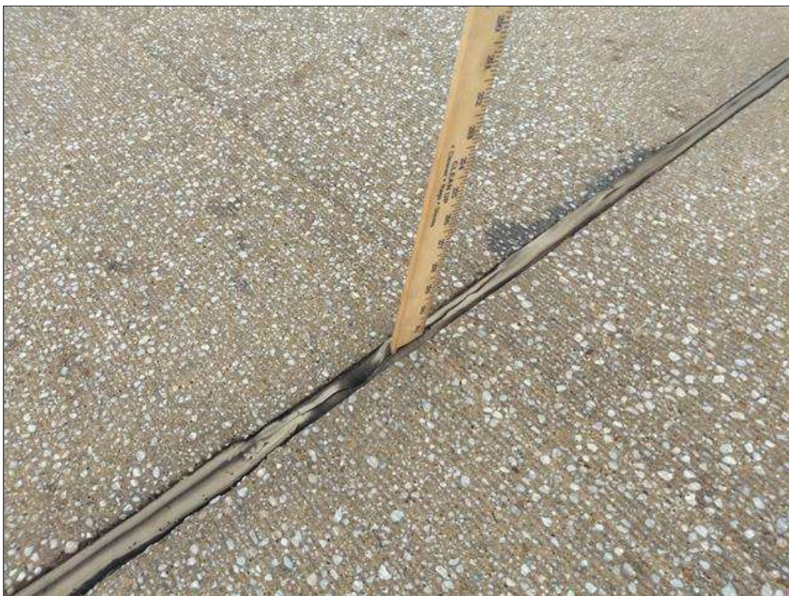
Span 89 Expansion Joint Bent 88: SCATTERED THROUGHOUT BOTH LANES, SEAL DAMAGED AND TORN (25 FEET)
