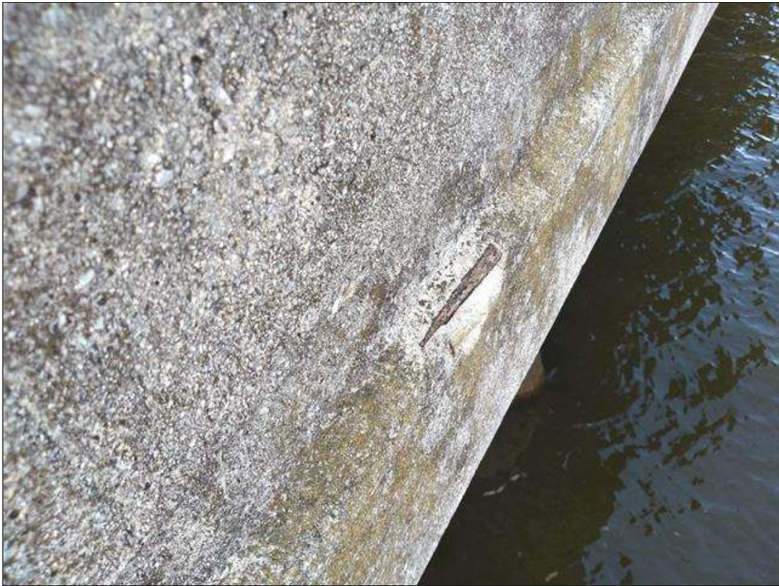
Span 16 Left Bridge Rail: 2 SPALLS ON BACK OF RAIL UP TO 3 INCH LONG X 1 INCH HIGH X 1 INCH DEEP WITH EXPOSED REINFORCEMENT AT BENT 15 AND 10 FEET FROM BENT 15.
