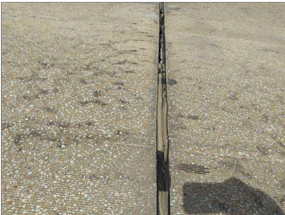
Span 67 Expansion Joint Bent 66: BOTH LANES AND SHOULDERS, SEAL DAMAGE ( UP TO FULL LENGTH)
