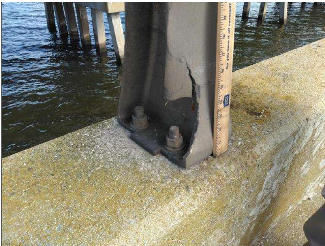
Span 34 Left Bridge Rail: (PAR) RAIL POST 6, IMPACT DAMAGE
