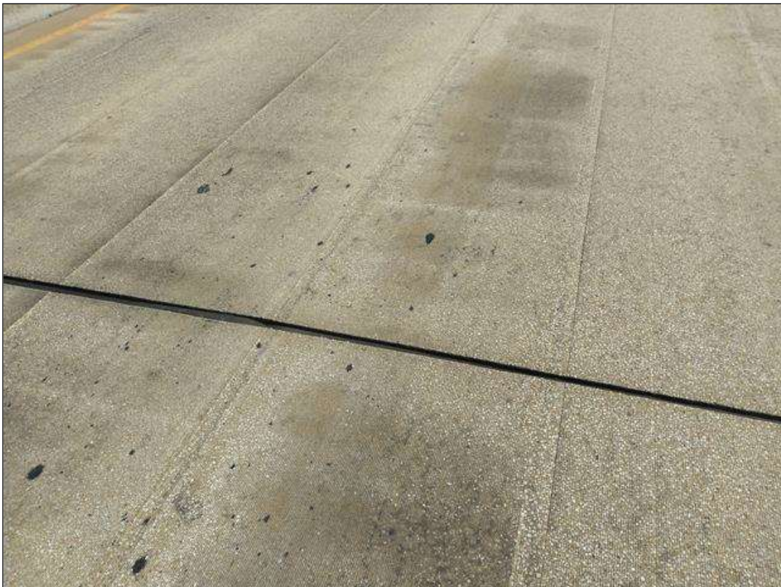
Span 118 Expansion Joint Bent 117: RIGHT LANE NEAR CENTERLINE OF ROADWAY, SPALL (6INCHES X2INCHES X 1/2 INCHES) (NOT FOUND 9/13/22)
