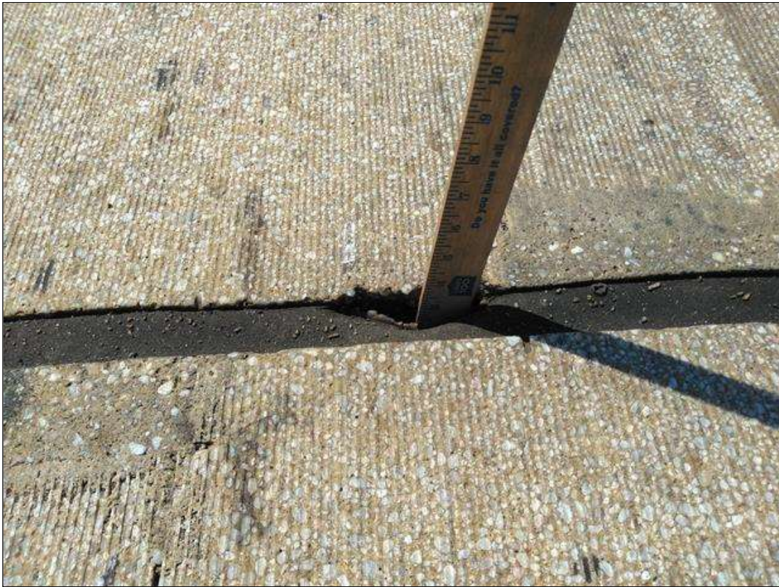
Span 179 Expansion Joint Bent 178: AT BENT 178, RIGHT LANE 5 INCH WIDE X 1 INCH LONG SPALL WITH NO JOINT SEAL ADHESION
