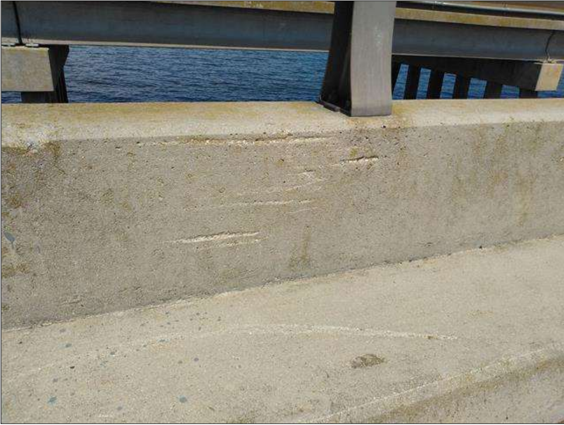
Span 50 Left Bridge Rail: RAIL AT RAILPOST 2, IMPACT SPALLS (4) UP TO 2 FEET LONG X 0.50 INCH DEEP
