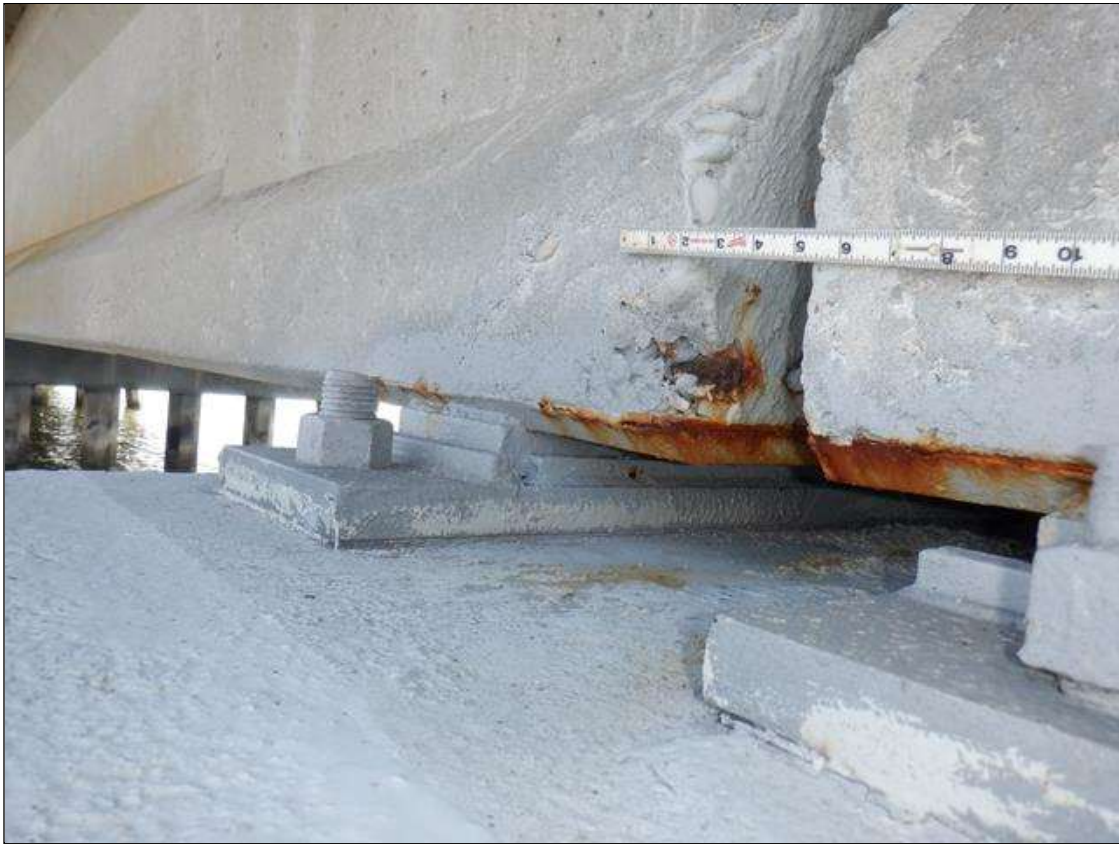
Span 9 Beam 1: NORTH FACE OF BOTTOM FLANGE, AT BENT 8, SPALL (5INCHES X 3INCHES X 2 INCHES) WITH EXPOSED RUSTED STRANDS
