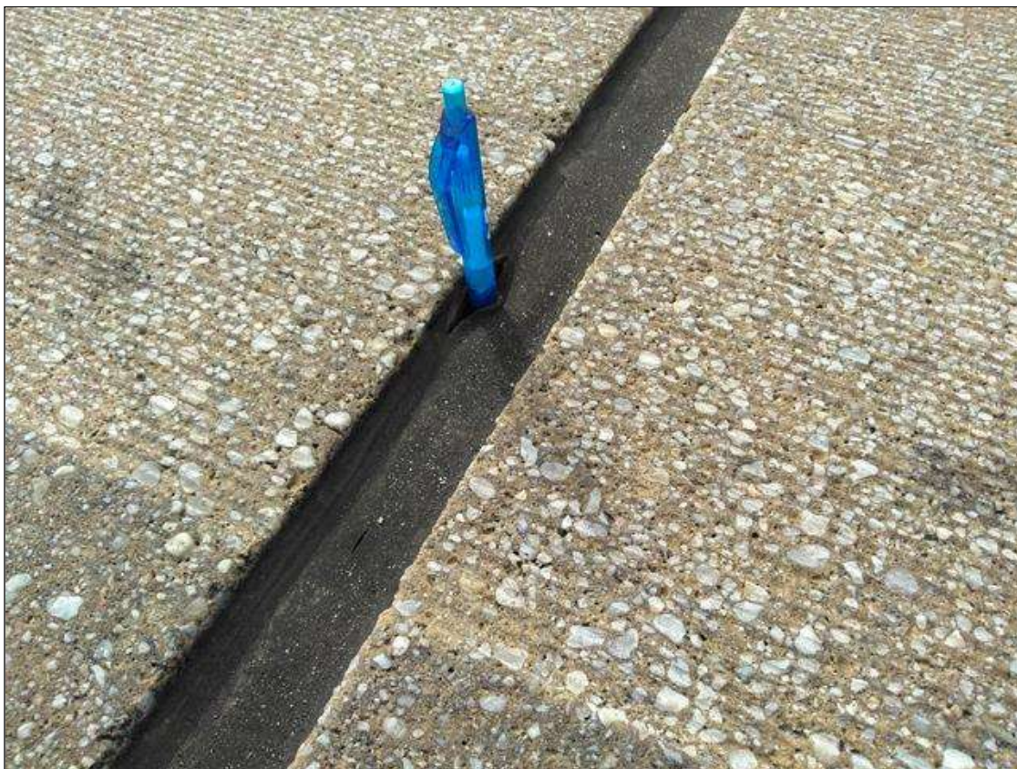
Span 113 Expansion Joint Bent 112: AT BENT 112, INTERMITTENT THROUGHOUT MULTIPLE CRACKS UP TO 3 INCHES LONG
