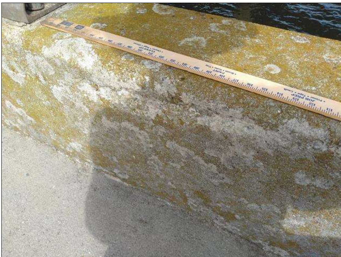
Span 30 Left Bridge Rail: RAIL AT RAILPOST 2, IMPACT SPALL (2FEET X 3INCHES X 1INCH)
