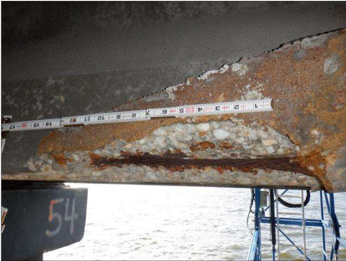
Span 54 Beam 3: (PAR) NORTH FACE OF BOTTOM FLANGE AT 9 FEET FROM BENT 54, SPALL (2 FEET X 9 INCHES X UP TO 3 INCHES) WITH (2) EXPOSED RUSTED STRANDS, SECTION LOSS (20 PERCENT)
