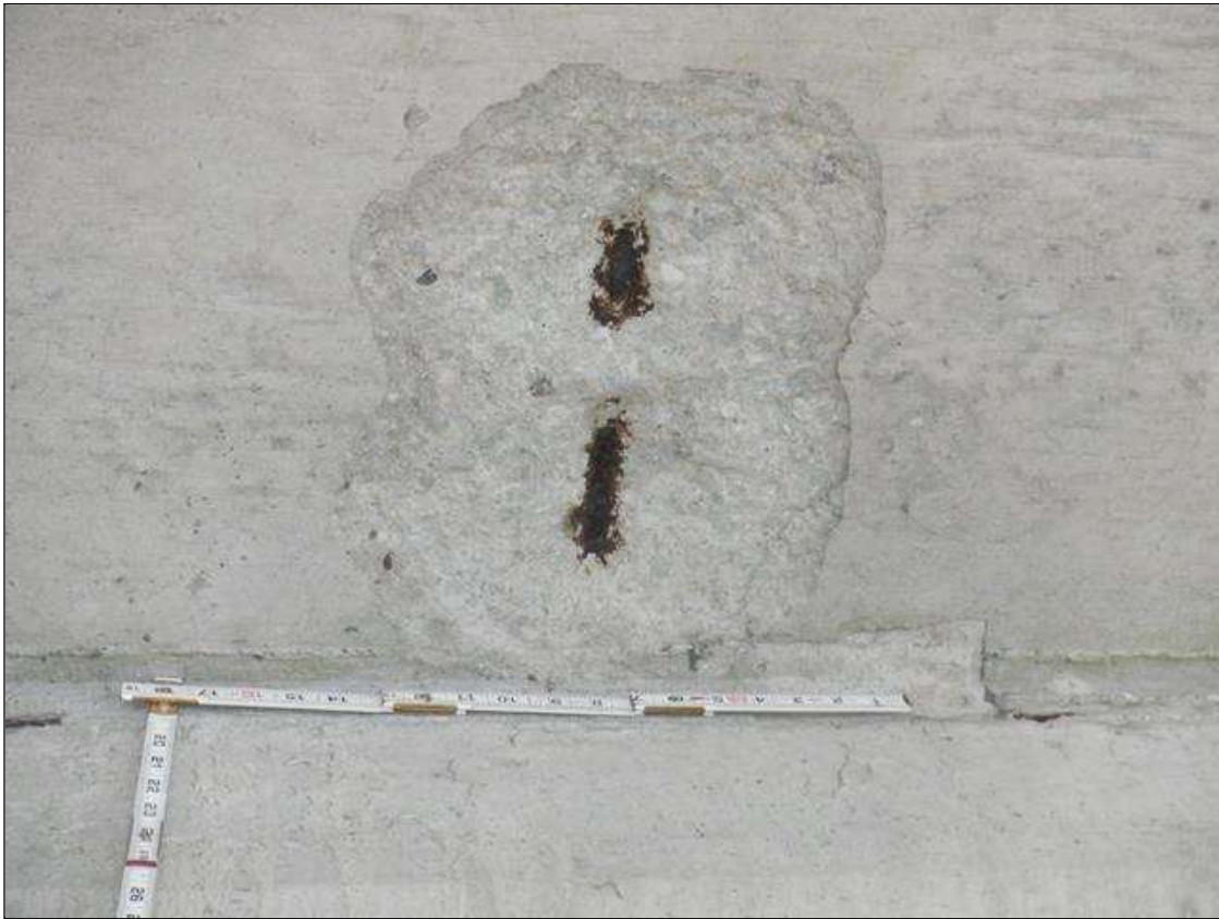
Span 44 Deck: UNDERSIDE OF DECK, BAY 2 NEXT TO BEAM 3 AT 7 FEET FROM BENT 44, SPALL (15 INCHES X 12 INCHES X 1/2 INCHES) WITH EXPOSED RUSTED REBAR
