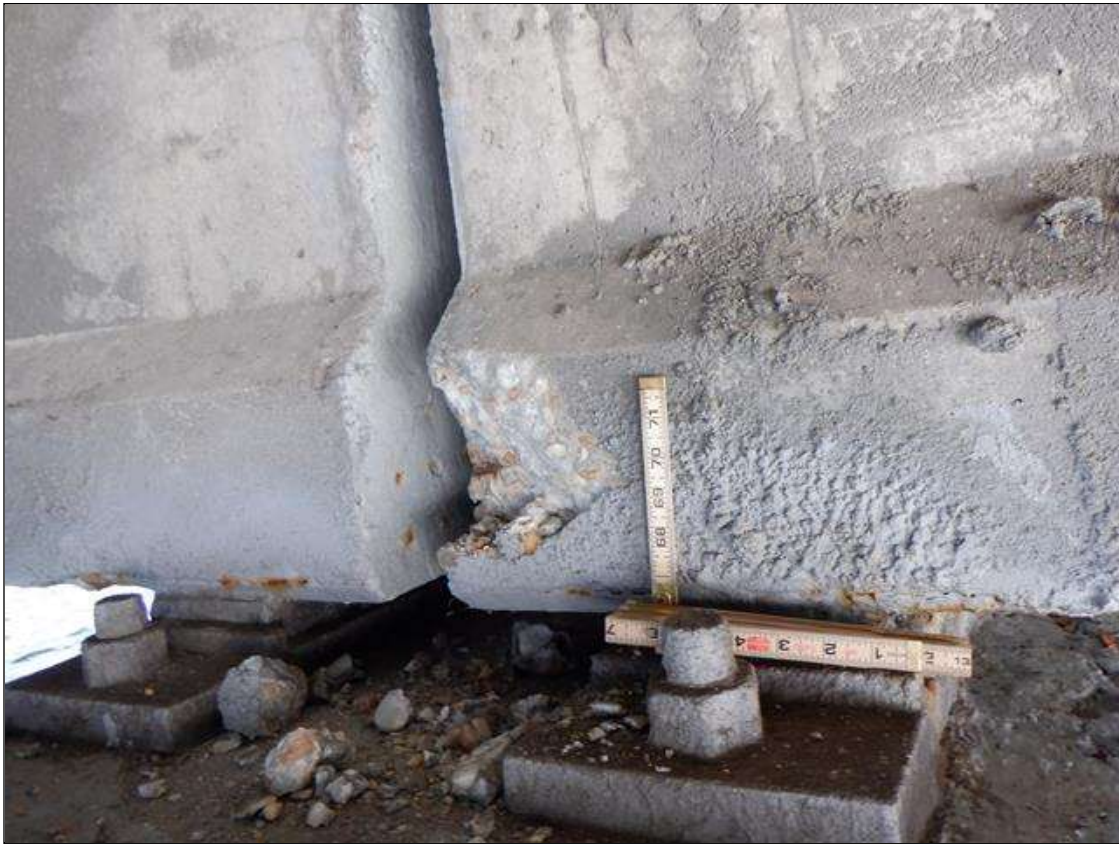
Span 118 Beam 3: (PAR) BOTTOM FLANGE SOUTH FACE AT BENT 117, SPALL (6 INCHES LONG X 6 INCHES HIGH X 1.5 INCHES DEEP) WITH (1) ON EXPOSED RUSTED STRAND (NO LOSS)
