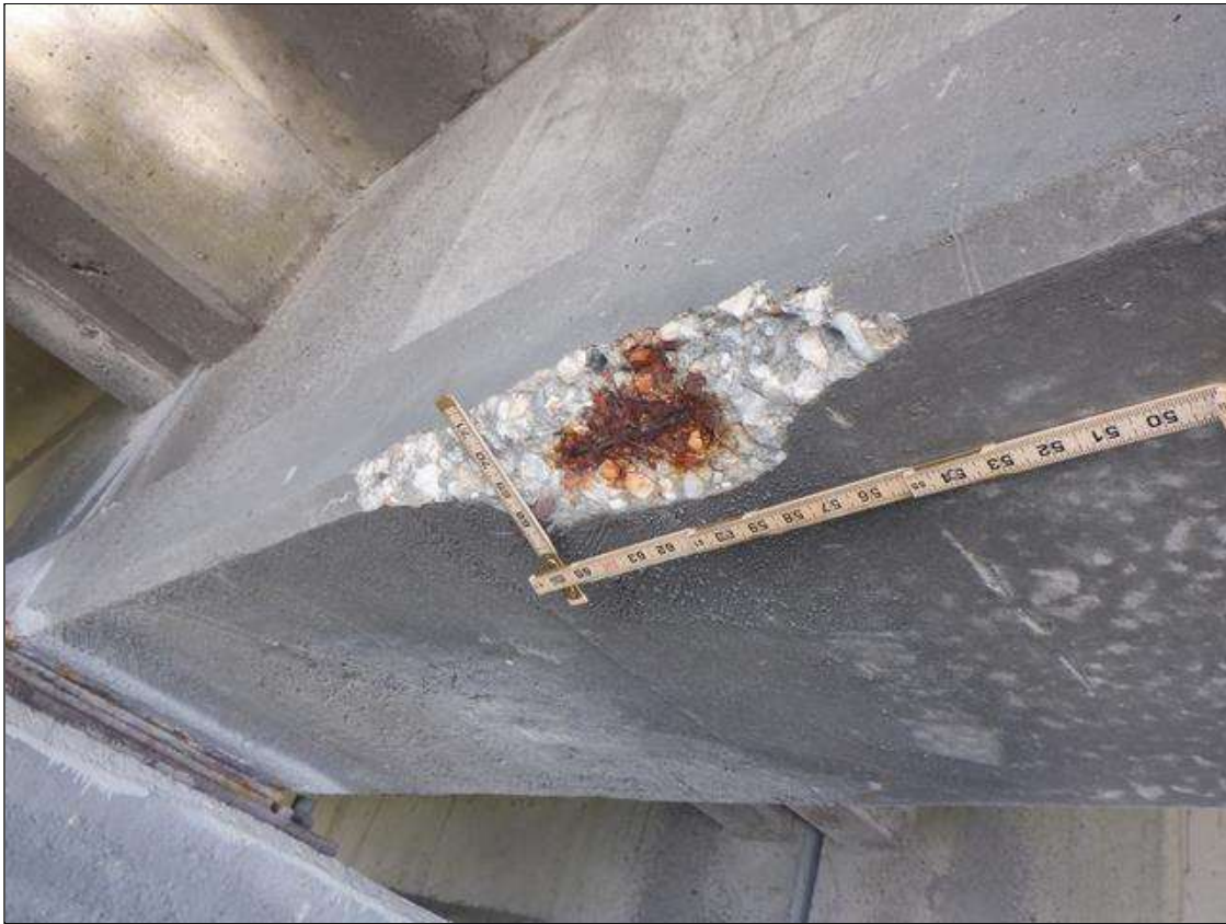
Span 122 Beam 2: (PAR) SOUTH FACE OF BOTTOM FLANGE AT 8 FEET FROM BENT 121, SPALL (16 INCHES LONG X 3 INCHES HIGH X 4 INCHES WIDE X 1.5 INCHES DEEP) WITH (1) EXPOSED RUSTED STRAND (10 PERCENT SECTION LOSS)
