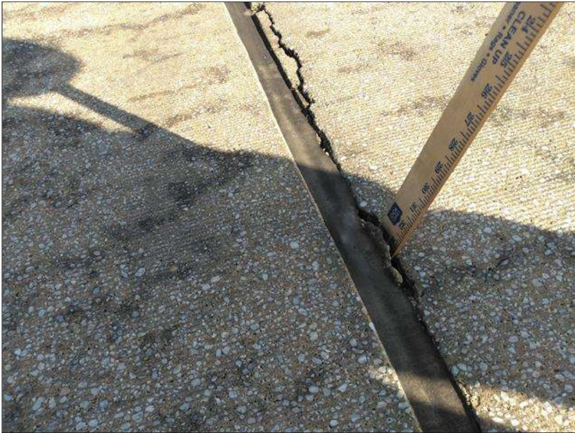
Span 213 Expansion Joint Bent 212: AT BENT 212, EDGD SPALLING IN RIGHT LANE ALONG JOINT, UP TO 7 FEET X 4 INCHES X PARTIAL DEPTH)
