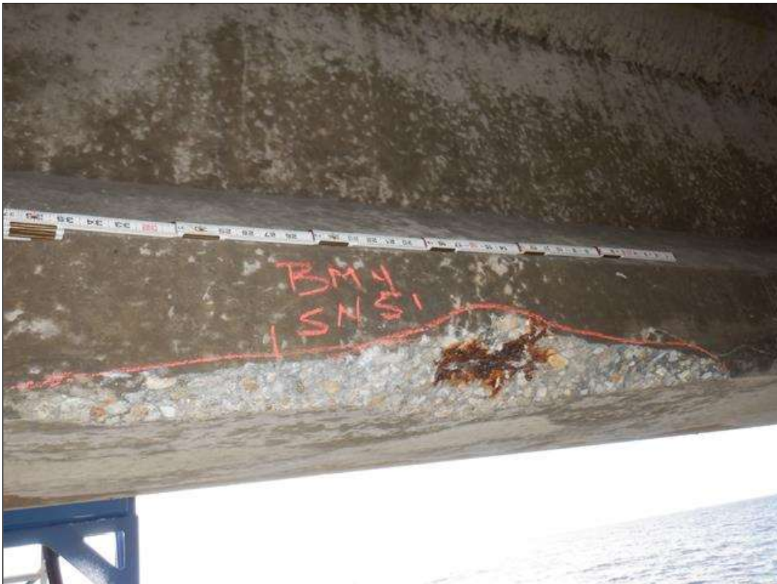
Span 51 Beam 4: (PAR) BOTTOM FLANGE NORTH FACE, 10 FEET FROM BENT 51, SPALL (36 INCHES LONG X 4 INCHES HIGH X 2 INCHES DEEP) WITH EXPOSED RUSTED STRANDS (10 PERCENT SECTION LOSS)
