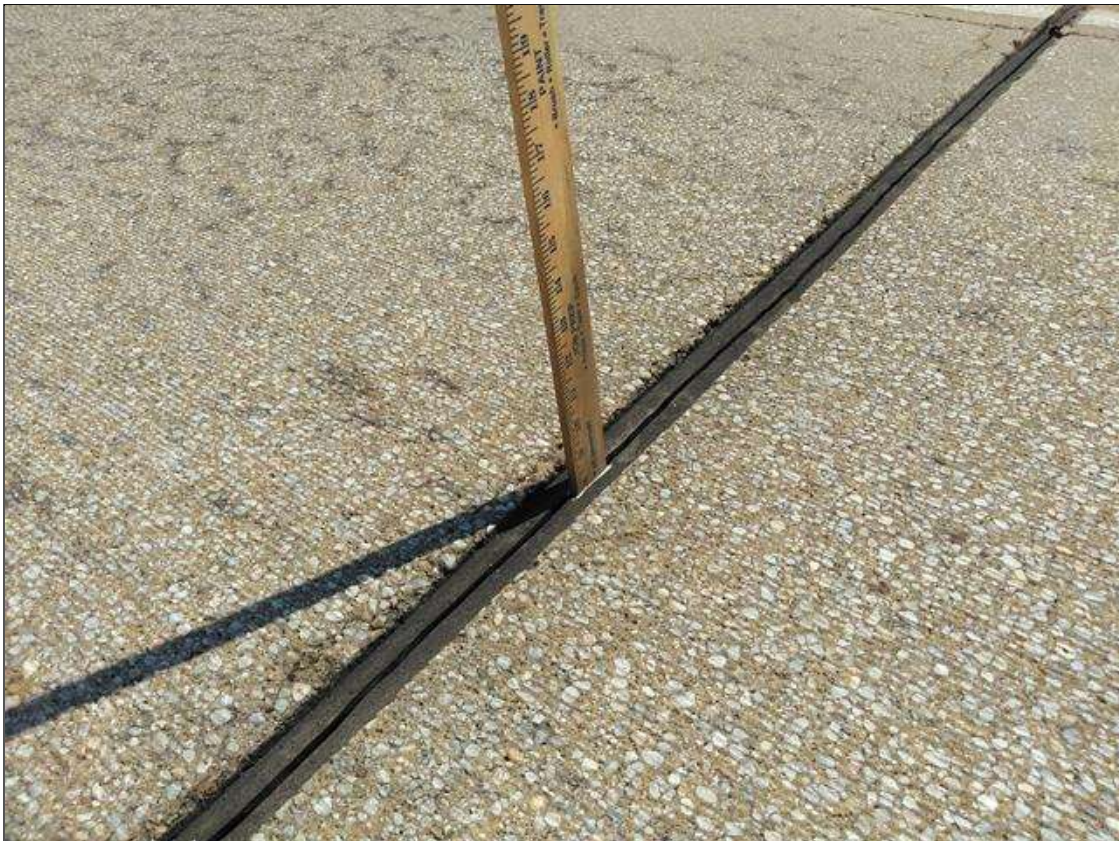
Span 171 Expansion Joint Bent 170: AT BENT 170, INTERMITTENT FULL DEPTH CRACKING THROUGHOUT
