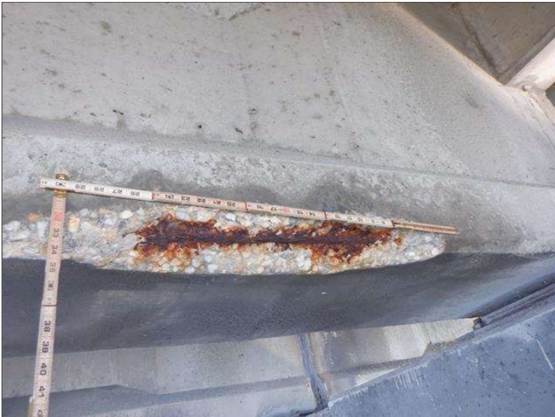
Span 216 Beam 2: (PAR) SOUTH FACE OF BOTTOM FLANGE, AT 4 FEET FROM BENT 216, SPALL (32 INCHES X 6 INCHES X 2 INCHES) WITH EXPOSED STRAND (10 PERCENT SECTION LOSS) ON STRAND
