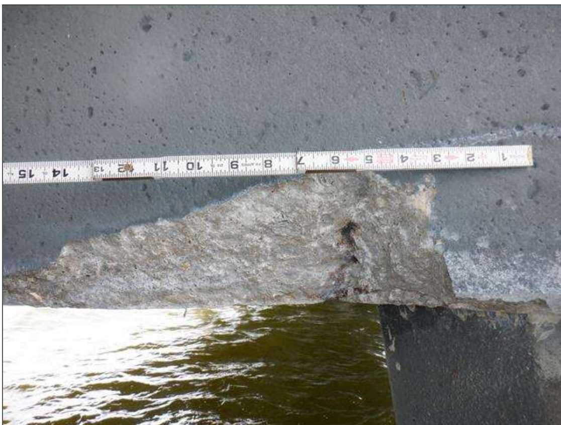
Bent 58 Cap 1: WEST FACE UNDER BEAM 2, SPALL (24 INCHES LONG X 8 INCHES HIGH)
