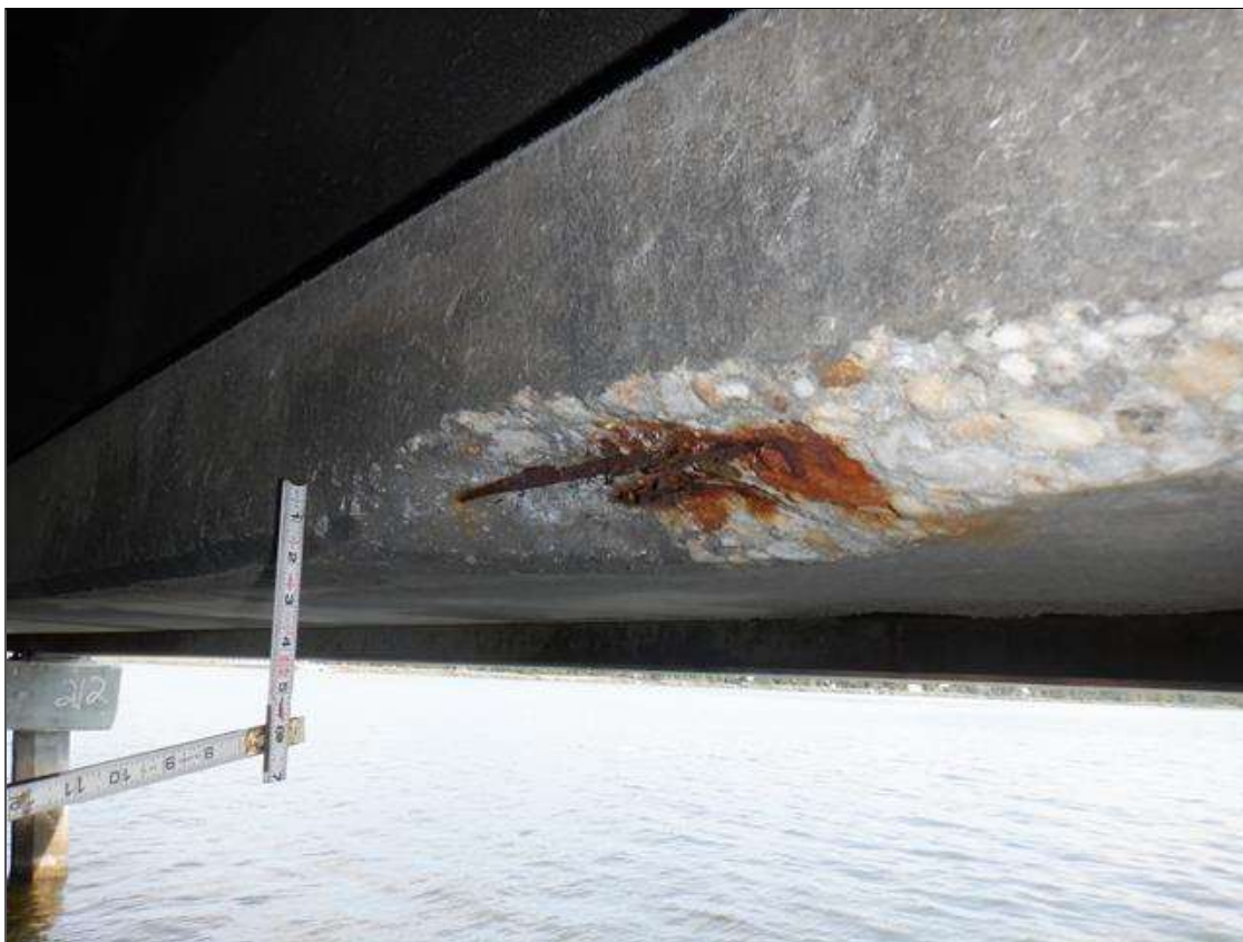
Span 212 Beam 3: (PAR) NORTH FACE OF BOTTOM FLANGE AT 13FEET FROM BENT 211, SPALL (21 INCHES X 8 INCHES X 2 INCHES) WITH (2) EXPOSED RUSTED STRANDS (75 PERCENT SECTION LOSS) ON BOTTOM LEFT STRAND AT FAILED PATCHED AREA
