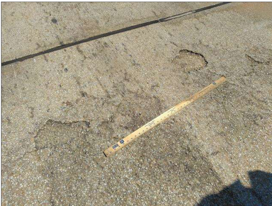
Span 178 Deck: RIGHT LANE AT 2FEET FROM BENT 178, (2) SPALLS (UP TO 8INCHES DIAMETER X 1/2INCHES)
