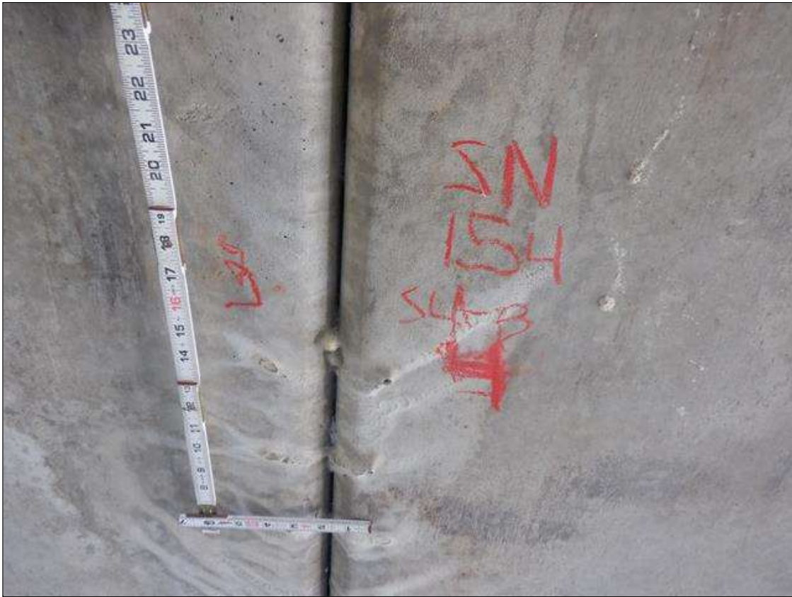
Span 154 Slab 3: BETWEEN SLABS 3 AND 4, MULTIPLE AREAS OF EFFLORESCENCE
