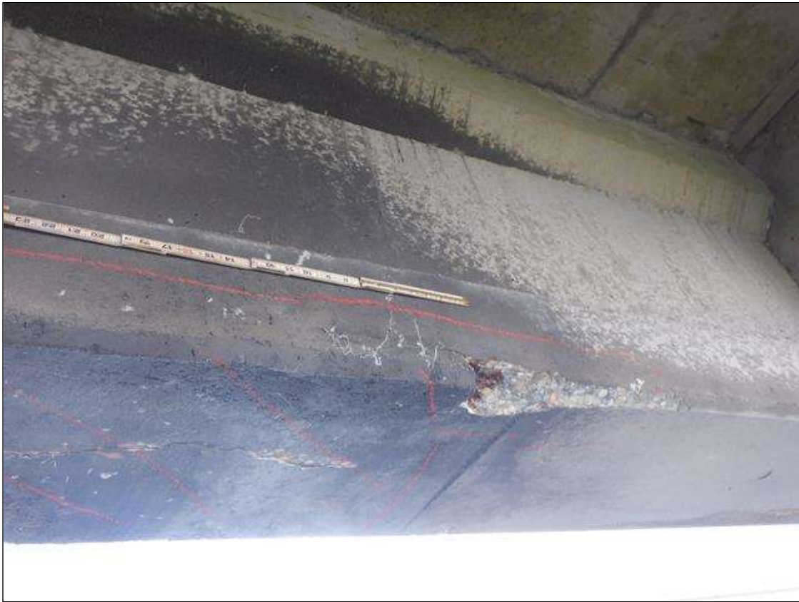
Span 104 Beam 3: (PAR) NORTH FACE OF BOTTOM FLANGE NEAR MIDSPAN, SPALL (40INCHES X 3INCHES X 12 INCHES ON BOTTOM X 2 INCHES DEEP) WITH (2) EXPOSED RUSTED STRANDS
