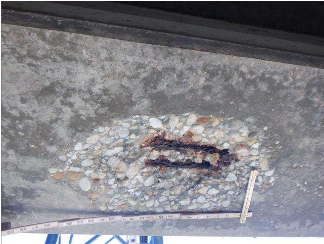
Span 112 Beam 4: (PAR) UNDERSIDE OF BOTTOM FLANGE 23 FEET FROM BENT 112, SPALL (20 INCHES LONG X 12 INCHES WIDE X 1 1/2 INCHES DEEP WITH (2) EXPOSED AND SEVERED STRANDS (10 PERCENT SECTION LOSS)
