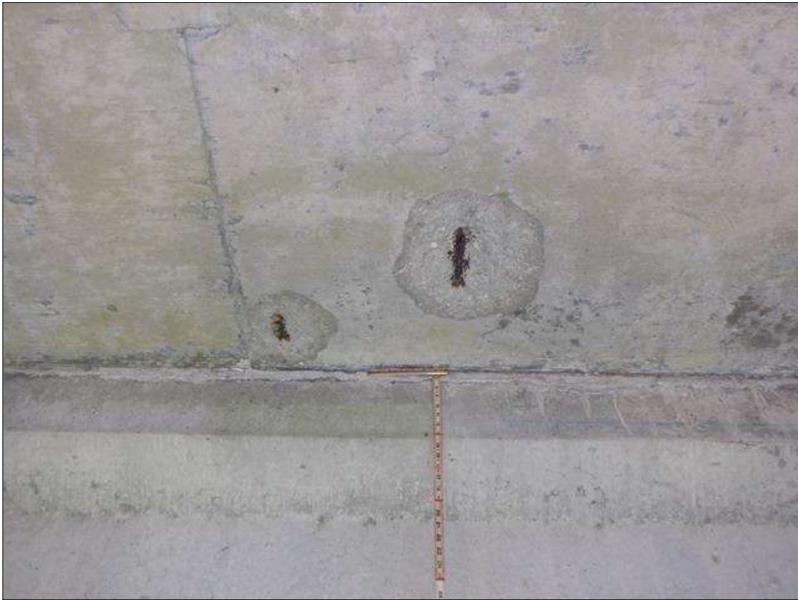
Span 117 Deck: UNDERSIDE OF DECK BAY 3 AT 16 FEET FROM BENT 117, (2) SPALLS (12 INCHES X 12 INCHES X 1 INCHES) WITH EXPOSED RUSTED REBAR
