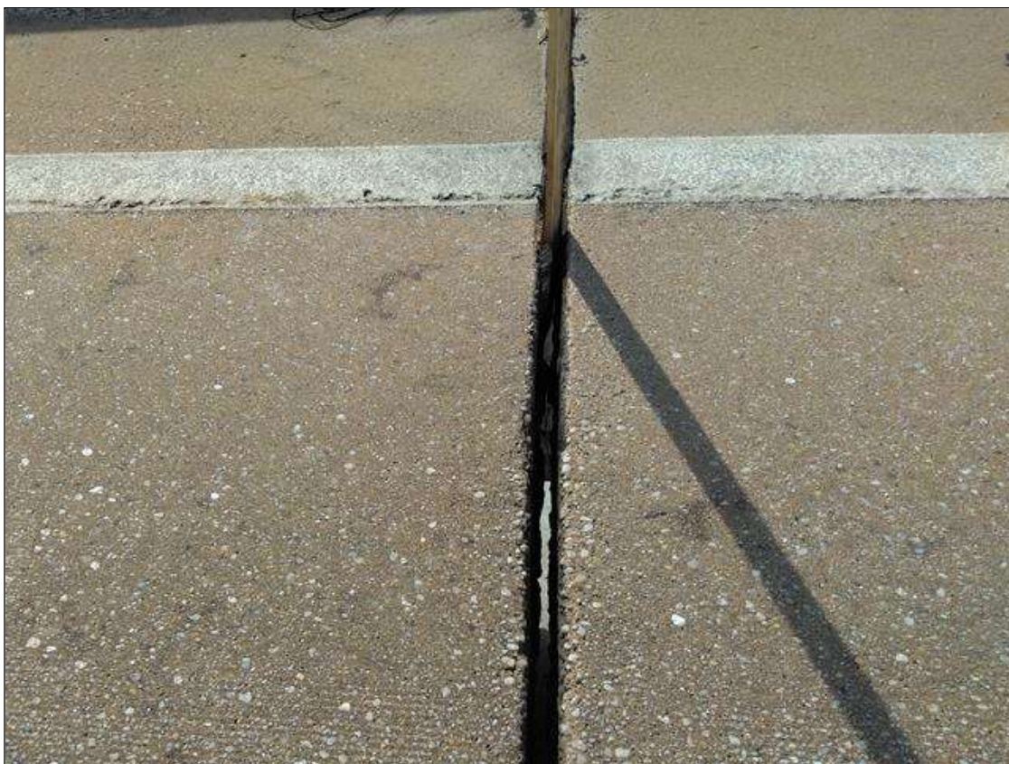
Span 131 Expansion Joint Bent 130: FULL WIDTH CRACKED, TORN, OR MISSING
