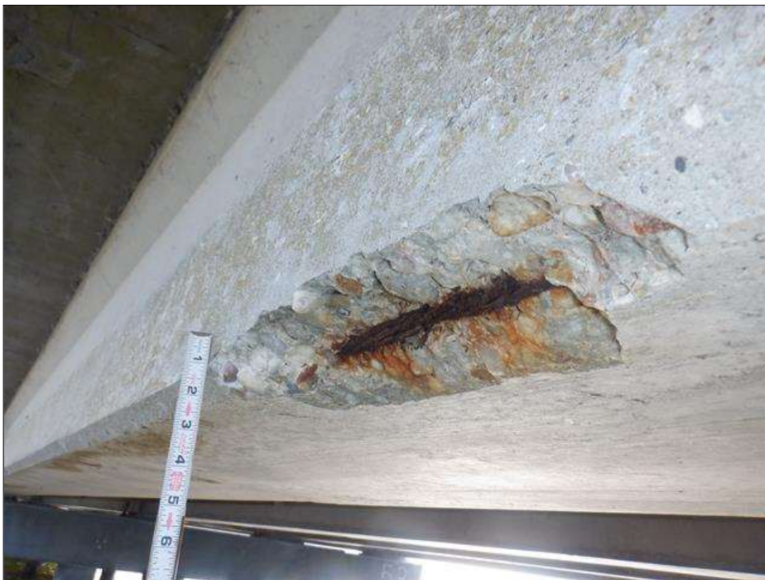
Span 53 Beam 1: (PAR) NORTH FACE OF BOTTOM FLANGE, AT 22FEET FROM BENT 52, SPALL (15INCHES X 4INCHES X 2 INCHES) WITH EXPOSED RUSTED STRAND, SECTION LOSS (20 PERCENT)
