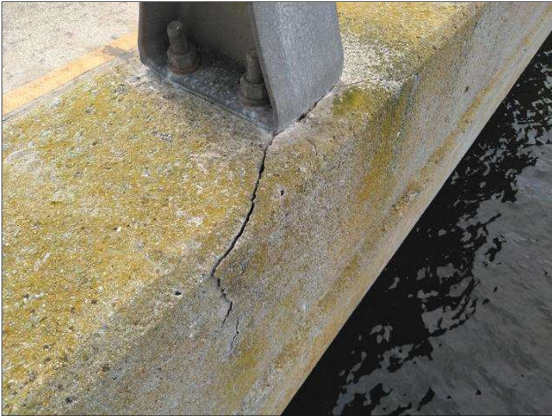
Span 68 Left Bridge Rail: DELAMINATION AT BACK OF RAILING AT POST 4, 16 INCH LONG X 9 INCHES HIGH
