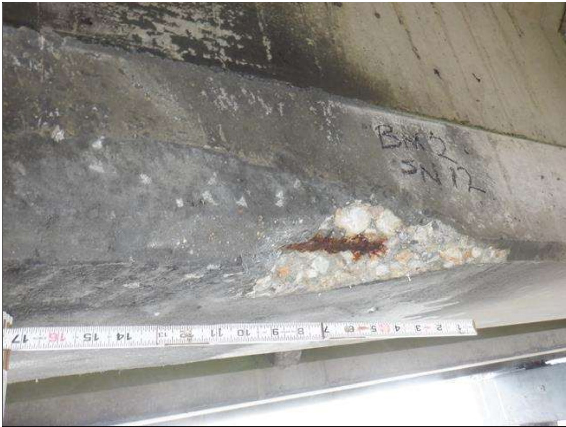
Span 12 Beam 2: (PAR) BOTH FACES OF BOTTOM FLANGE AT 23 FEET FROM BENT 11, (2) PATCHED AREAS (UP TO 30 INCHES X 12 INCHES), WITH SPALL (12 INCHES X 3 INCHES X 3 INCHES DEEP) WITH EXPOSED RUSTED STRANDS (20 PERCENT SECTION LOSS)
