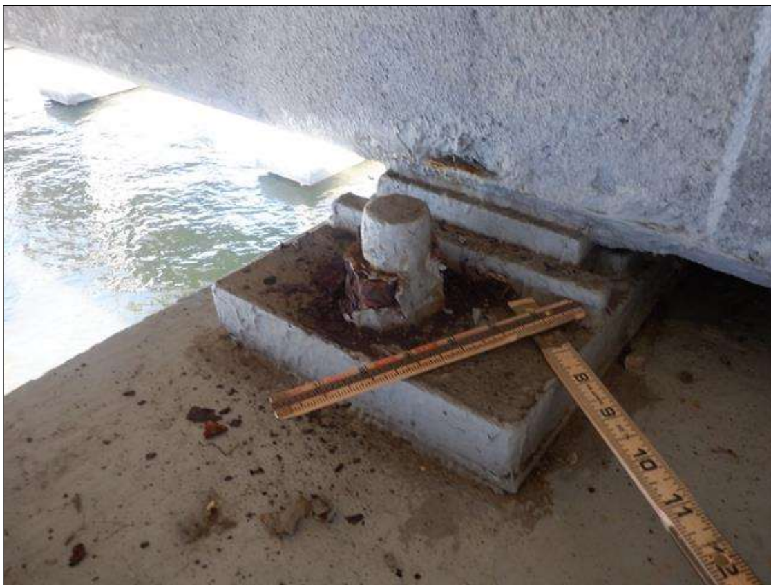
Span 182 Beam 2 - Far Bearing: SOUTH ANCHOR BOLT NUT, 25 PERCENT SECTION LOSS, AT BENT 182
