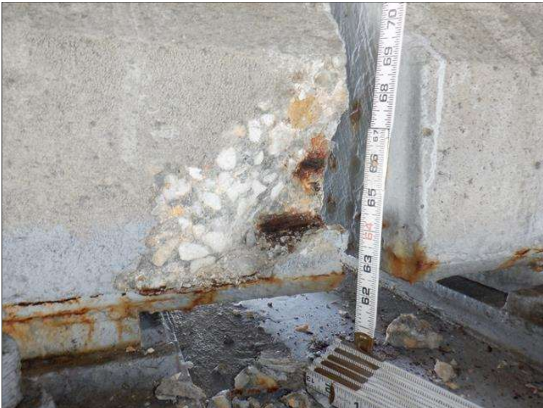
Span 207 Beam 1: SOUTH FACE OF BOTTOM FLANGE AT BENT 207, SPALL (6 INCHES X 6 INCHES X 2 INCHES DEEP) WITH EXPOSED RUSTED REINFORCING (NO MEASURABLE LOSS)
