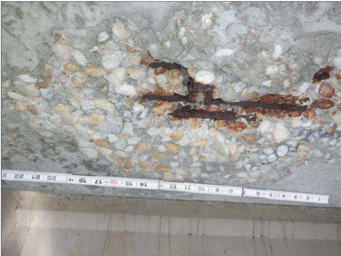
Span 99 Beam 4: (PAR) UNDERSIDE OF BOTTOM FLANGE AT 23 FEET FROM BENT 98, SPALL (21 INCHES X 11 INCHES X UP TO 2 INCHES) WITH EXPOSED STRANDS WITH (20 PERCENT SECTION LOSS) ON STRANDS
