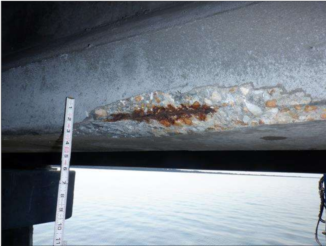
Span 155 Beam 4: (PAR) BOTTOM FLANGE NORTH FACE AT 10 FEET FROM BENT 155, SPALL (18 INCHES LONG X 5 INCHES HIGH X 1.5 INCHES DEEP) WITH EXPOSED RUSTED STRANDS (10 PERCENT SECTION LOSS)
