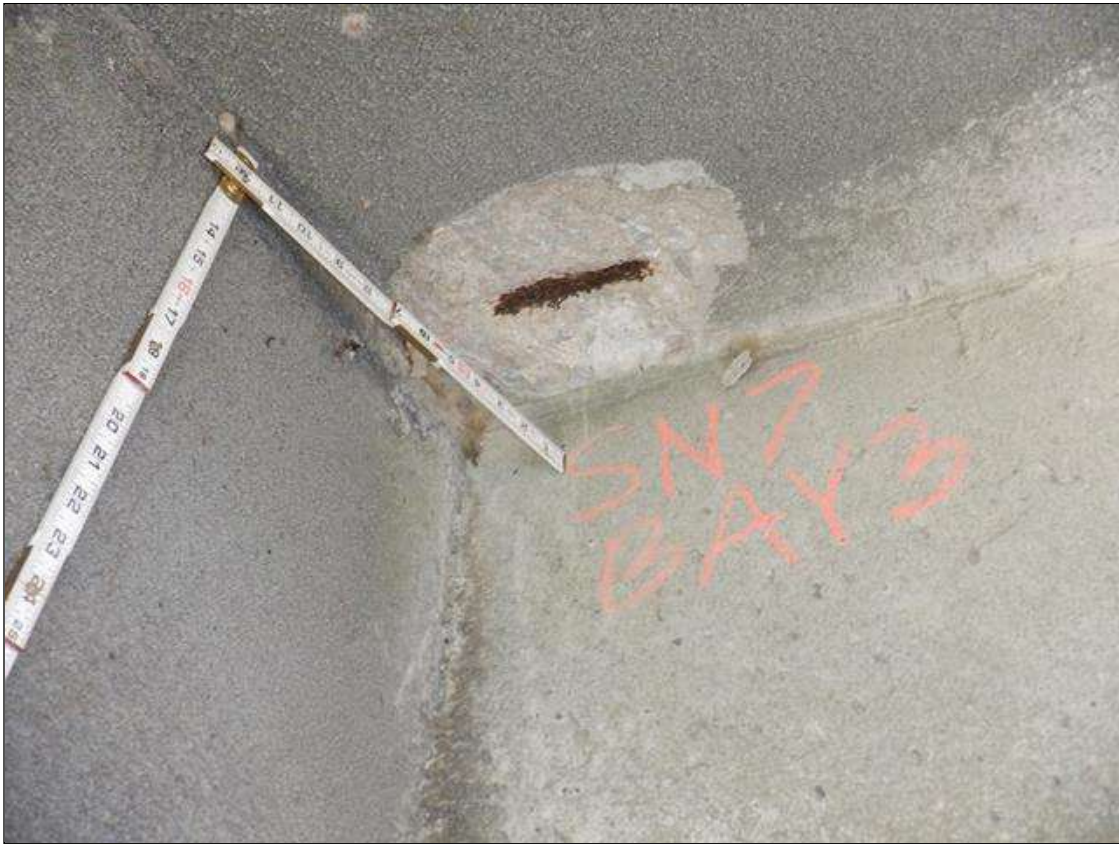
Span 7 Deck: UNDERSIDE OF DECK AT BENT 6 BAY 3, SPALL (8 INCH DIAMETER X 1 INCH DEEP) WITH EXPOSED RUSTED REINFORCING (10 PERCENT SECTION LOSS)
