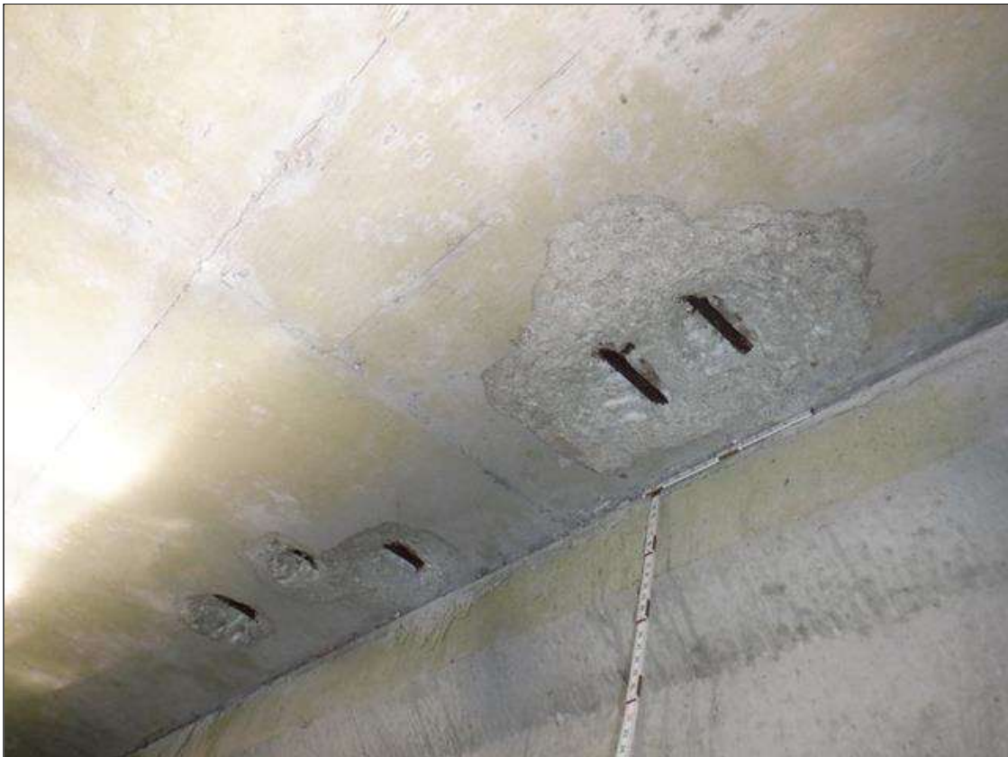
Span 45 Deck: UNDERSIDE OF DECK, BAY 3 NEXT TO BEAM 4, AT 10 FEET FROM BENT 45, (4) SPALLS (UP TO 2 FEET X 18 INCHES X UP TO 2 INCHES) WITH EXPOSED RUSTED REBAR
