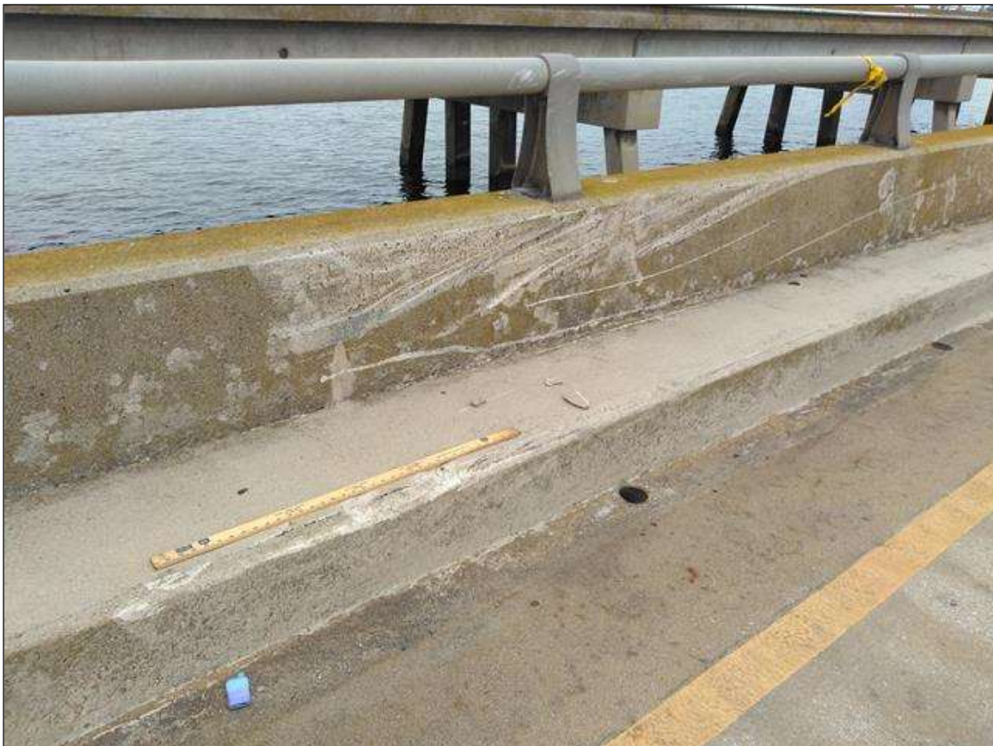
Span 83 Left Bridge Rail: BETWEEN POSTS 2 AND 4, IMPACT SCRAPES ON RAIL AND SPALLS ON CURB UP TO 3 FEET LONG X 3 INCHES HIGH X 1 INCH DEEP
