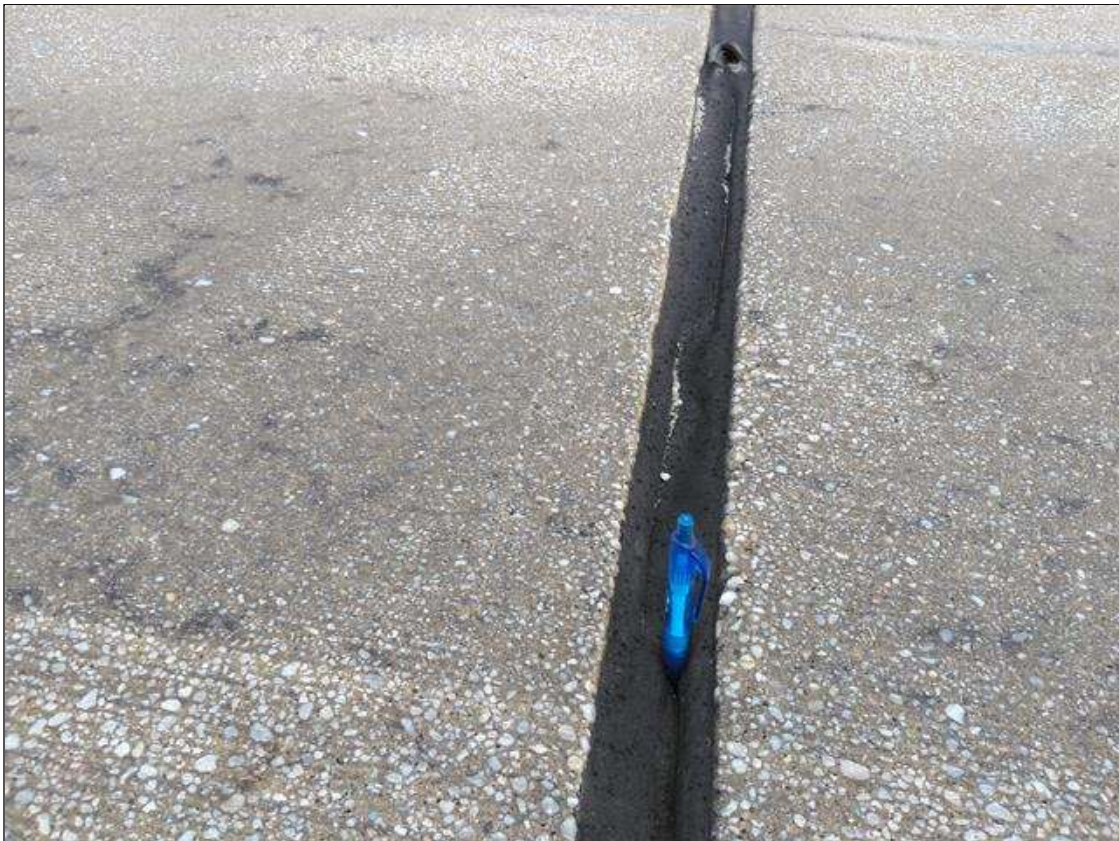
Span 115 Expansion Joint Bent 114: SEAL DAMAGE. FULL DEPTH CRACK FULL WIDTH
