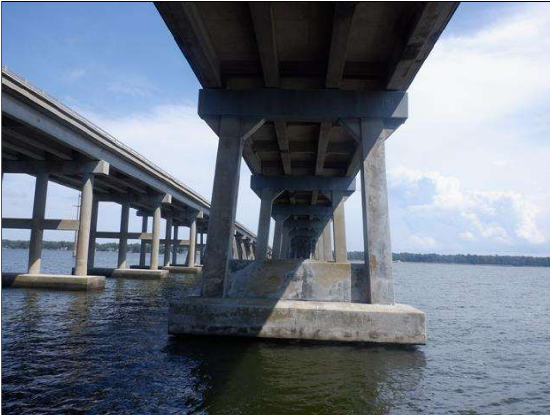
TYPICAL INTERIOR BENT PROFILE, TWO PILES IN VIEW
