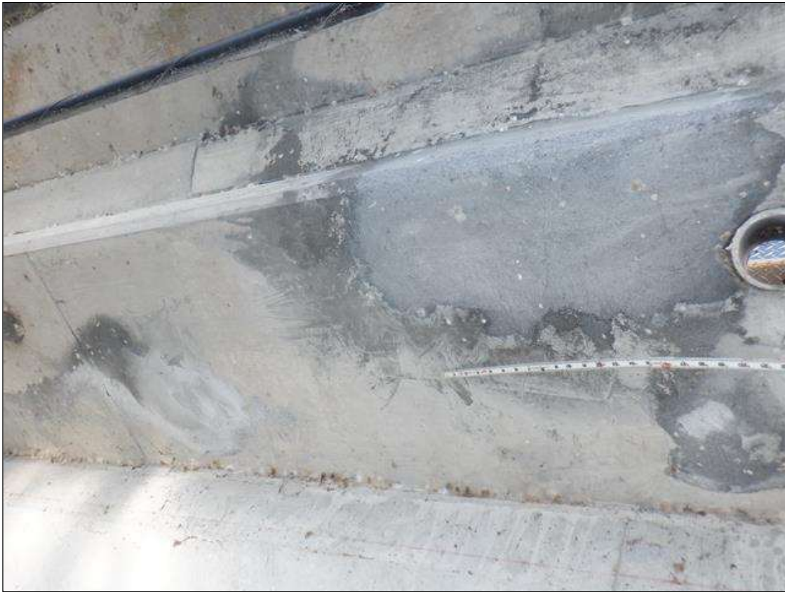
Span 4 Deck: UNDERSIDE OF DECK, SOUTH OVERHANG AT 20 FEET FROM BENT 3, 2 (TWO) PATCHED AREAS (UP TO 24 INCHES X UP TO 18 INCHES)
