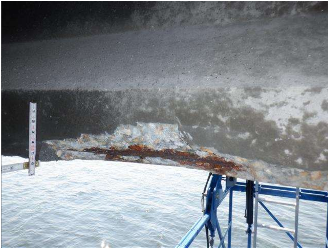
Span 159 Beam 4: (PAR) BOTTOM FLANGE NORTH FACE AT 12 FEET FROM BENT 159, FAILED PATCH/SPALL (32 INCHES LONG X 4 INCHES HIGH X UP TO 2 INCHES DEEP) WITH EXPOSED RUSTED STRANDS (20 PERCENT SECTION LOSS)
