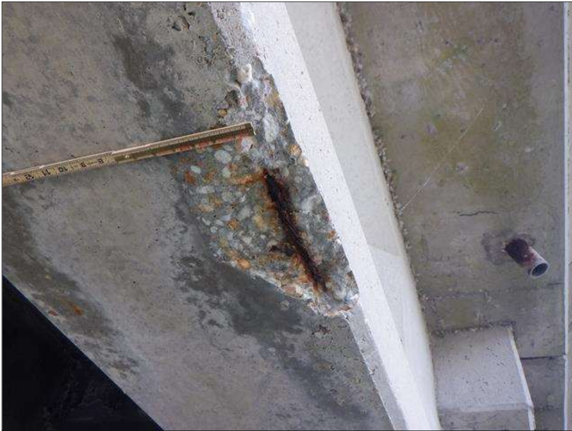
Span 122 Beam 1: (PAR) NORTH FACE OF BOTTOM FLANGE AT 6 FEET FROM BENT 121, SPALL (18 INCHES X 6 INCHES X 2 INCHES) WITH EXPOSED STRANDS (10 PERCENT SECTION LOSS) ON STRAND
