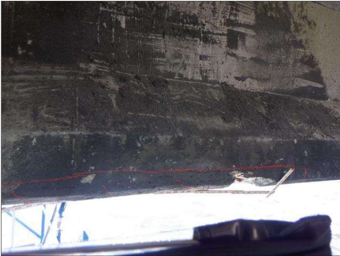
Span 103 Beam 4: (PAR) NORTH FACE OF BOTTOM FLANGE 25 FEET FROM BENT 103, DELAMINATION/SPALL (43 INCHES LONG X 4 INCHES HIGH X 8 INCHES ON BOTTOM FLANGE X 1 INCH DEEP WITH (1) EXPOSED REINFORCEMENT BAR (NO LOSS)
