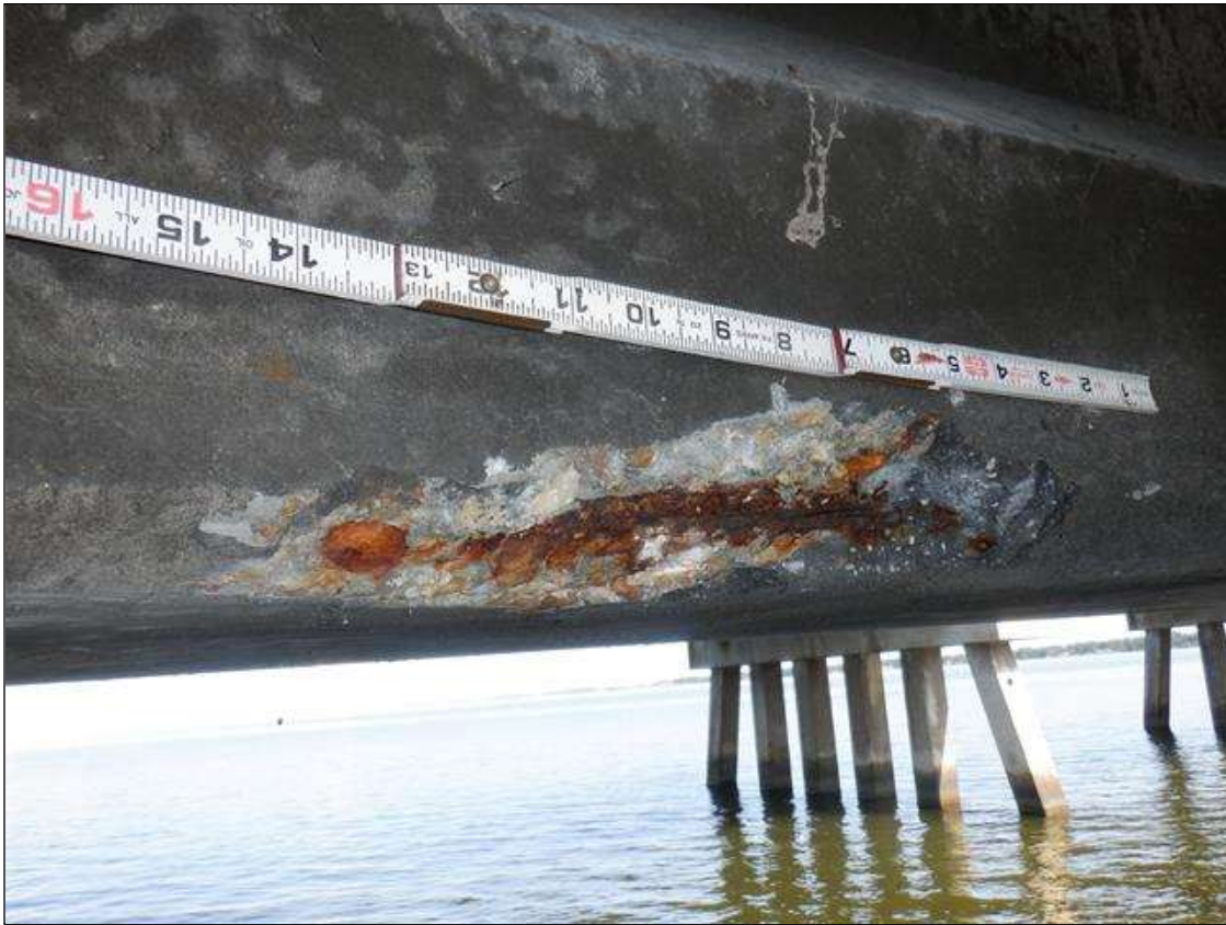
Span 160 Beam 1: (PAR) SOUTH FACE OF BOTTOM FLANGE AT 10 FEET FROM BENT 159, FAILED PATCH/SPALL (12 INCHES X 2 INCHES HIGH X 2 INCHES DEEP) WITH EXPOSED RUSTED STRANDS (10 PERCENT SECTION LOSS)
