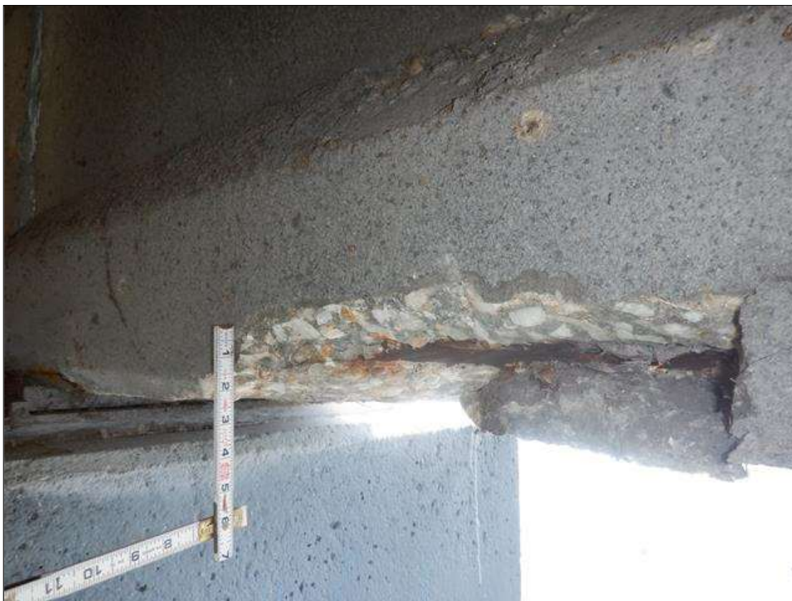
Span 100 Beam 4: (PAR) NORTH FACE BOTTOM FLANGE, AT 4 FEET FROM BENT 100, SPALL (19 INCHES X 10 INCHES X 2 INCHES) WITH EXPOSED STRANDS (5 PERCENT SECTION LOSS ON STRAND), DEBONDED (100 PERCENT LOSS)
