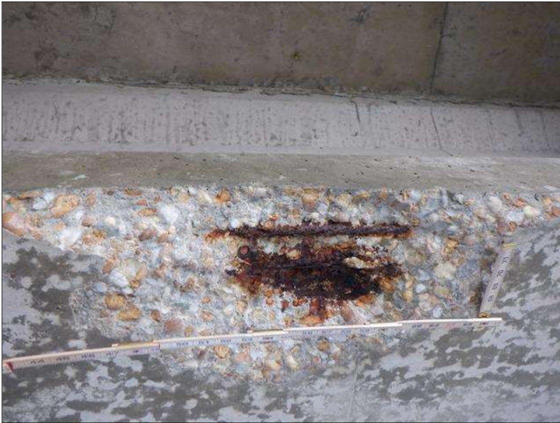
Span 139 Beam 2: (PAR) UNDERSIDE AND SOUTH FACE OF BOTTOM FLANGE AT 17 FEET FROM BENT 138, SPALL (30 INCHES X 12 INCHES X 2 INCHES) WITH (4) FOUR EXPOSED STRANDS (20 PERCENT SECTION LOSS) ON STRAND
