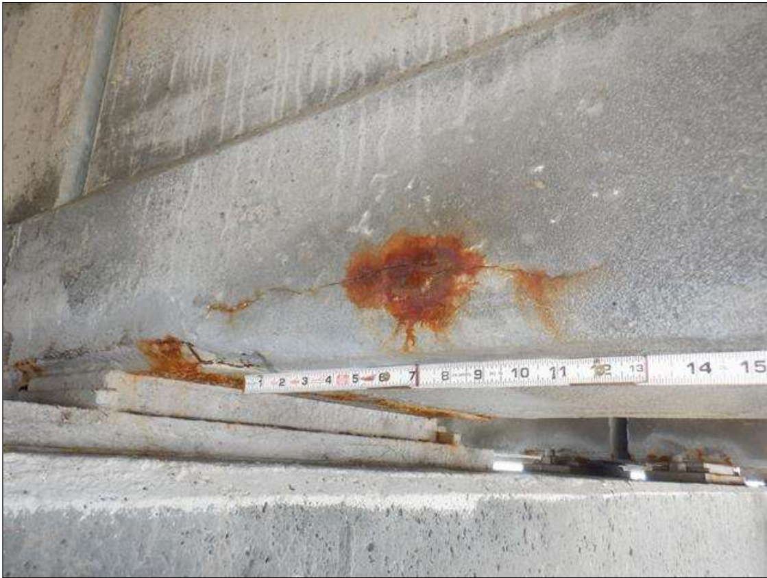
Span 68 Beam 2: NORTH FACE OF BOTTOM FLANGE AT BENT 68, HORIZONTAL CRACK (8 INCHES X 0.015 INCHES) WITH RUST STAIN
