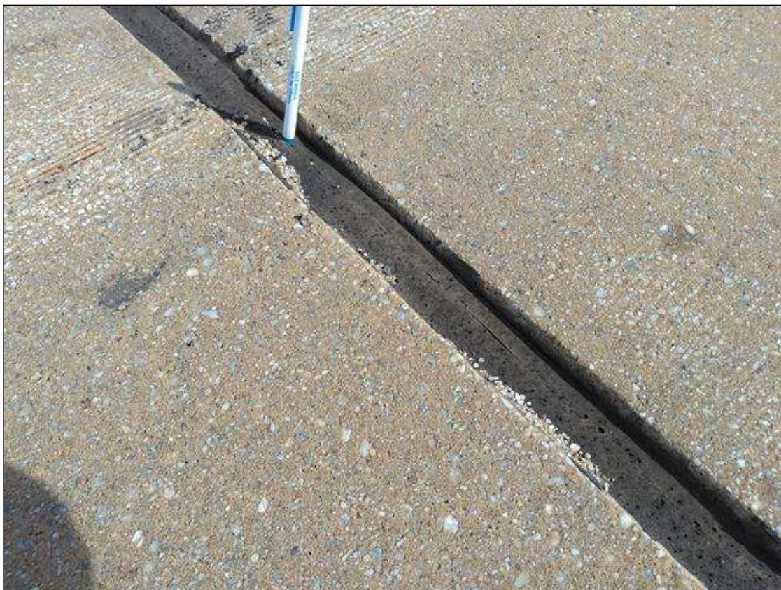
Span 232 Expansion Joint Bent 231: AT BENT 231, AT CENTER 2 FOOT LONG PARTIAL DEPTH CRACK
