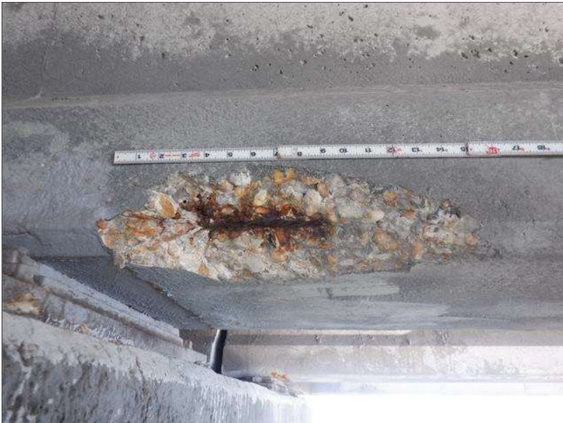
Span 166 Beam 3: (PAR) SOUTH FACE OF BOTTOM FLANGE AT 1FEET FROM BENT 165, SPALL (15 INCHES X 6 INCHES X 3 INCHES) WITH EXPOSED STRANDS (25 PERCENT SECTION LOSS) ON STRAND
