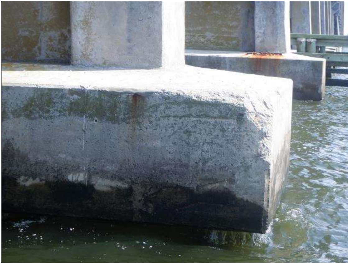
Bent 175 Footing: TOP WEST FACE NEAR SOUTH END, DELAMINATION (10 FEET X 1 FEET)
