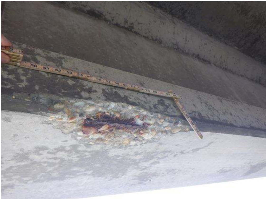
Span 148 Beam 4: (PAR) NORTH FACE OF BOTTOM FLANGE AT MIDSPAN, SPALL (16 INCHES X 4 INCHES X 2 INCHES) WITH EXPOSED STRANDS (5 PERCENT SECTION LOSS) ON STRAND
