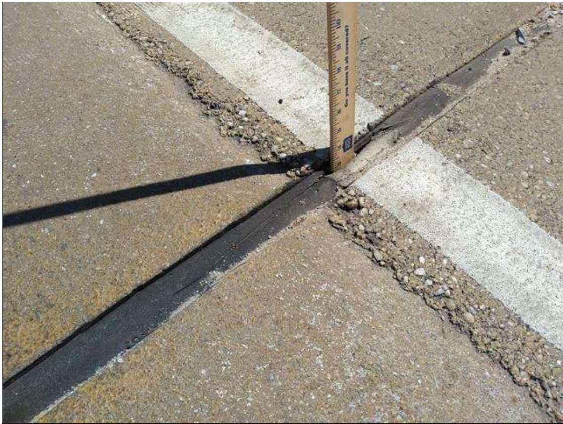
Span 51 Expansion Joint Bent 50: AT BENT 50, 2 CRACKS UP TO 1 FOOT LONG X FULL DEPTH AT CENTER AND RIGHT EDGE
