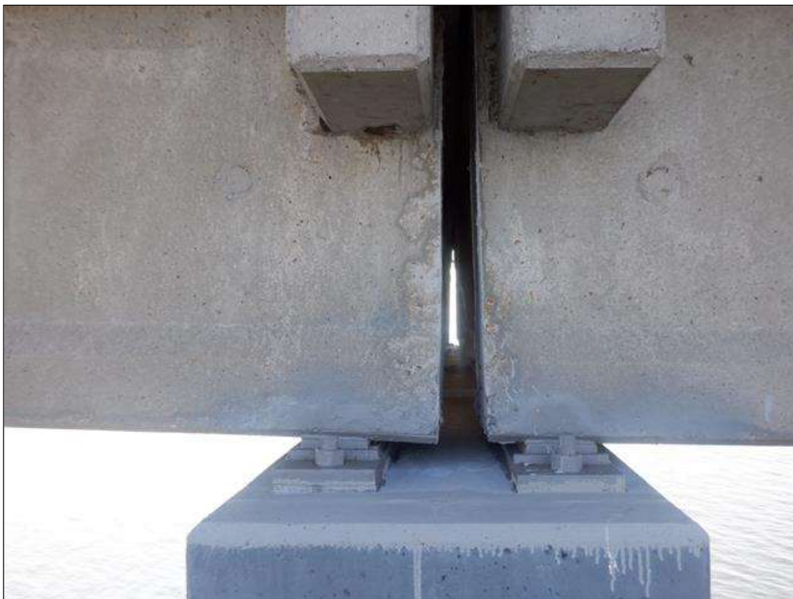
TYPICAL BEAM OVER INTERIOR BENT
