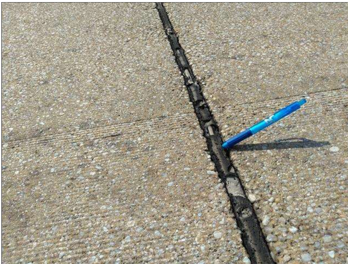
Span 126 Expansion Joint Bent 125: SCATTERED THROUGHOUT BOTH LANES, SEAL DAMAGED AND TORN (10 FEET)
