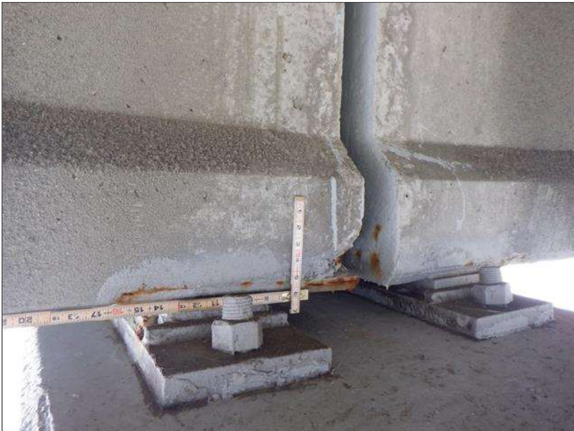
Span 143 Beam 2: (PAR) NORTH FACE OF BOTTOM FLANGE AT BENT 142, SPALL (3 INCHES X 2 INCHES X 2 INCHES) WITH EXPOSED STRANDS (5 PERCENT SECTION LOSS) ON STRAND
