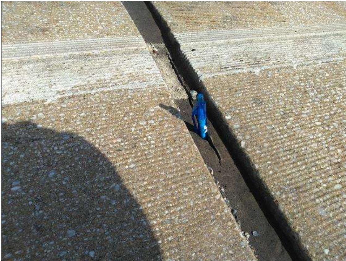
Span 125 Expansion Joint Bent 124: BENT 124, CRACK AT CENTERLINE 8 INCH LONG FULL DEPTH
