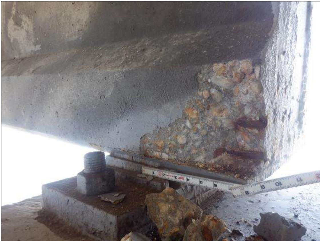
Span 173 Beam 4: (PAR) NORTH FACE AT BENT 172, SPALL (8 INCHES 6 INCHES X 2 INCHES DEEP) WITH TWO (2) EXPOSED STANDS (10 PERCENT LOSS)
