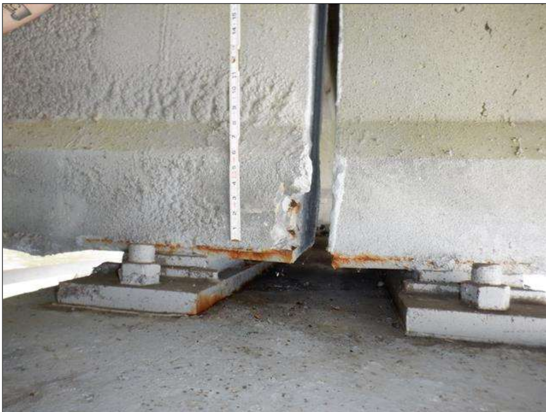
Span 1 Beam 3: SOUTH FACE OF BOTTOM FLANGE, AT BENT 1, SPALL (5 INCHES X 4 INCHES X 2 INCHES) WITH EXPOSED RUSTED PRESTRESSING
