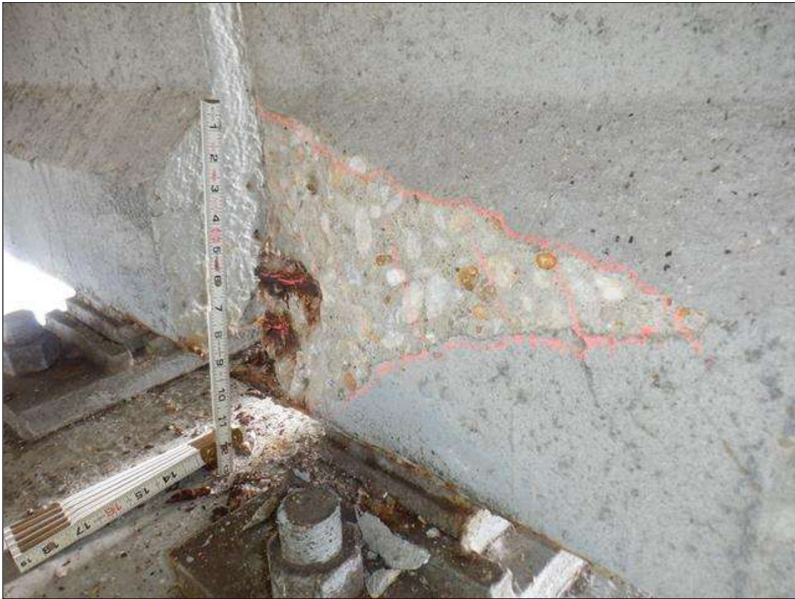
Span 38 Beam 4: (PAR) BOTTOM FLANGE NORTH FACE AT BENT 38, SPALL (16 INCHES LONG X 8 INCHES HIGH X UP TO 3 INCHES DEEP) WITH TWO (2) EXPOSED RUSTED STRANDS (5 PERCENT SECTION LOSS)
