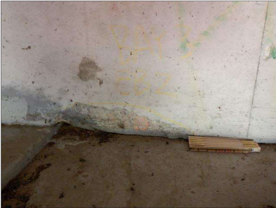
End Bent 2 Abutment: BAY 3 BACKWALL AT CAP, SPALL (18 INCHES LONG X 5 INCHES HIGH X 3 INCHES DEEP)
