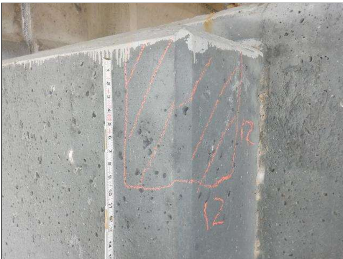
Bent 72 Cap 1: TOP OF A FRAME CAP SOUTHWEST CORNER OVER PILE 2, DELAMINATION (12 INCHES X 12 INCHES)
