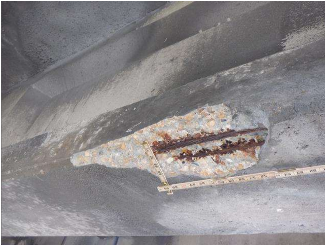
Span 137 Beam 2: (PAR) NORTH FACE OF BOTTOM FLANGE AT 10FEET FROM BENT 137, SPALL (20INCHES X 4INCHES X 2 INCHES) WITH (2) TWO EXPOSED AND SEVERED STRANDS (20 PERCENT SECTION LOSS)
