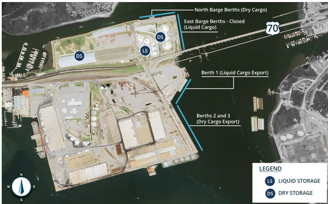
Figure 4. Without the Project, acid barges must navigate the narrow passage beneath the Newport River Bridge (US 70) to unload at Berth 1.
