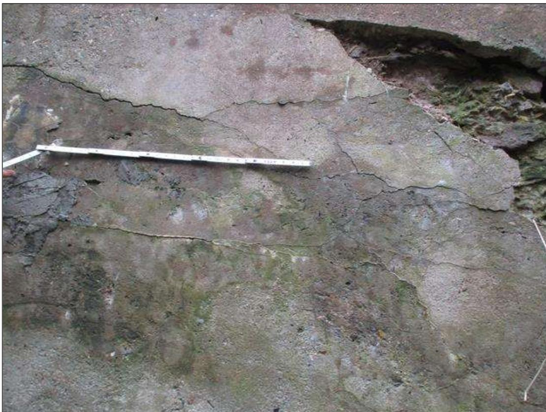
End Bent 2 Abutment: 15' OF UP TO 1/8" MAP CRACKING WITH EFFLORESCENCE IN FACE OF BREASTWALL IN VARIOUS LOCATIONS
