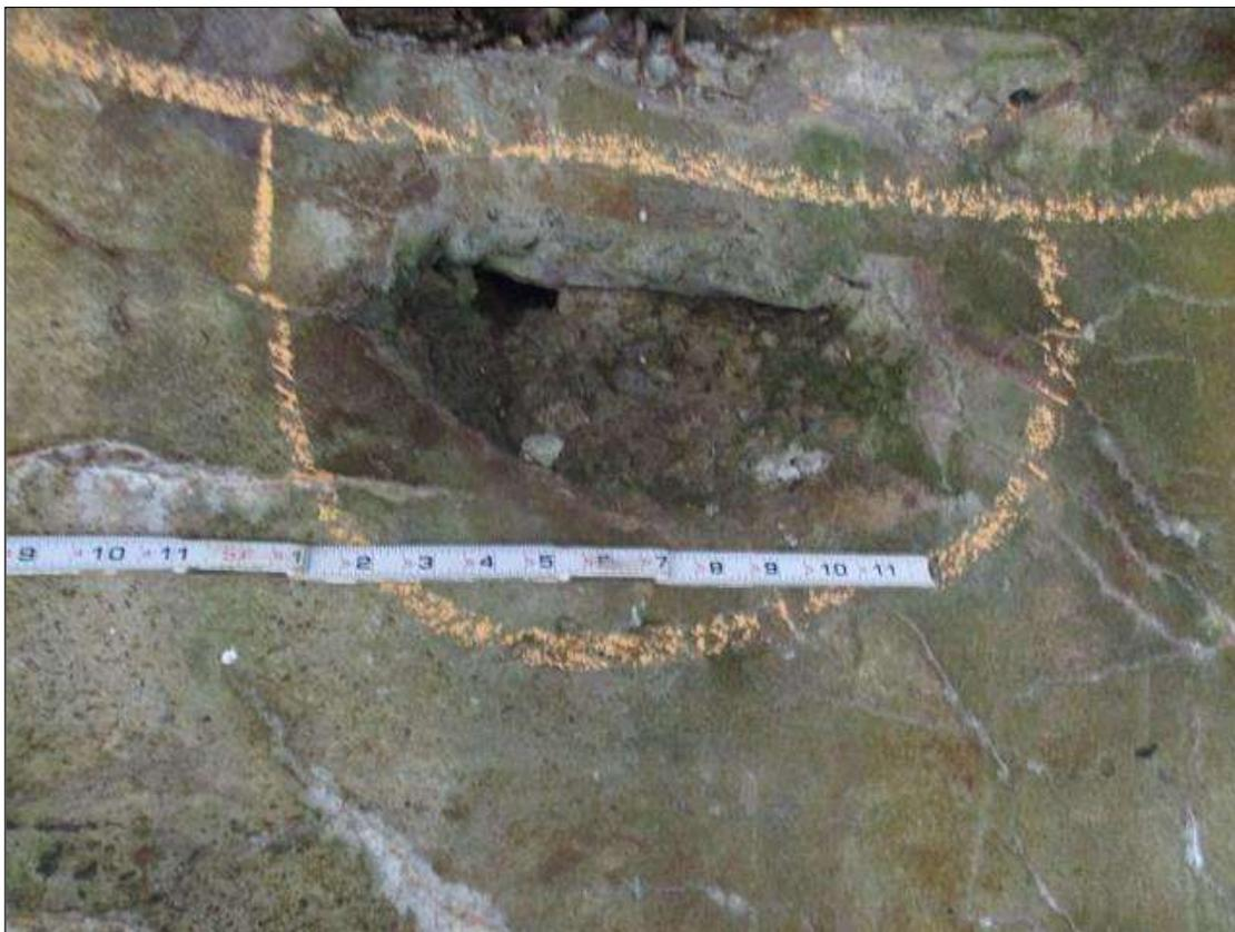
End Bent 1 Abutment: 10" X 5" X 1" DEEP SPALL IN FACE OF BREASTWALL BENEATH BAY 1 NEAR BOTTOM OF CAP
