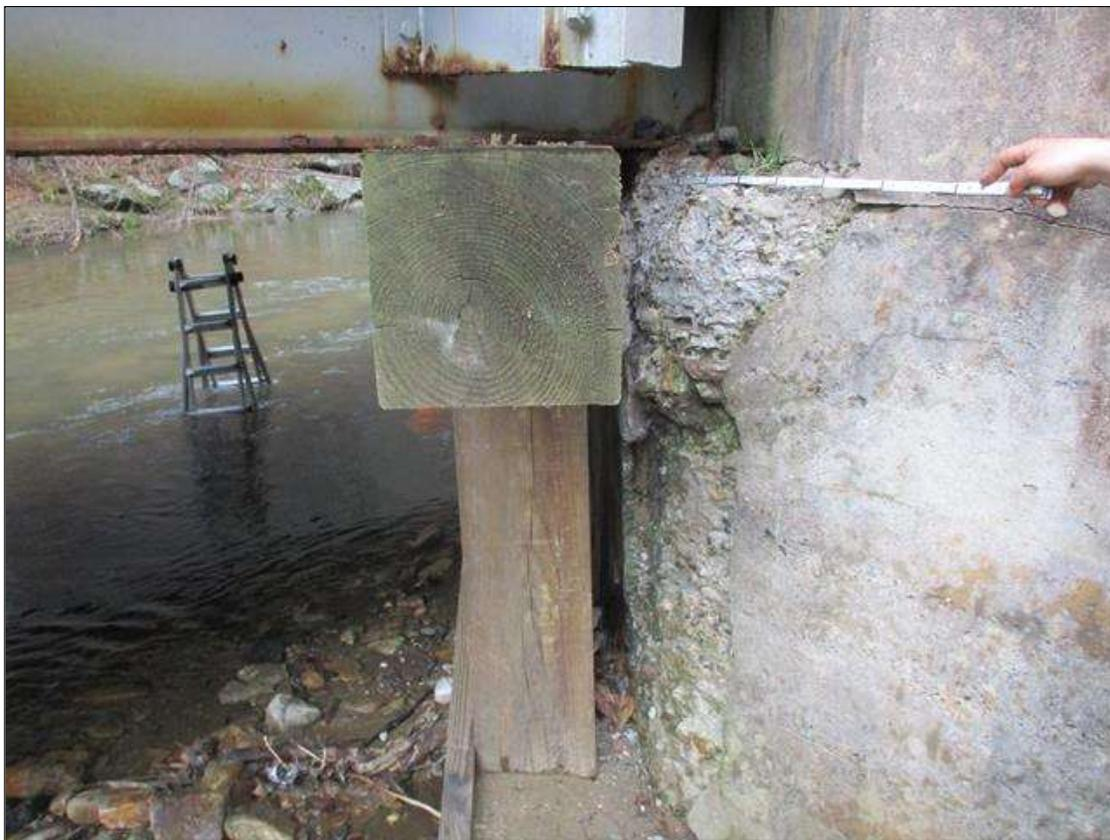
End Bent 2 Abutment: 36" LONG X 60" HIGH X UP TO 8" DEEP SPALL IN FACE OF BREASTWALL AT RIGHT END
