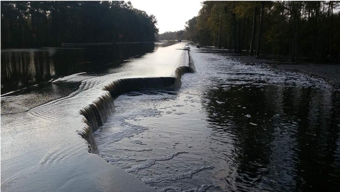
Figure 2.2B. Extensive Shoulder Damage following Hurricane Florence
