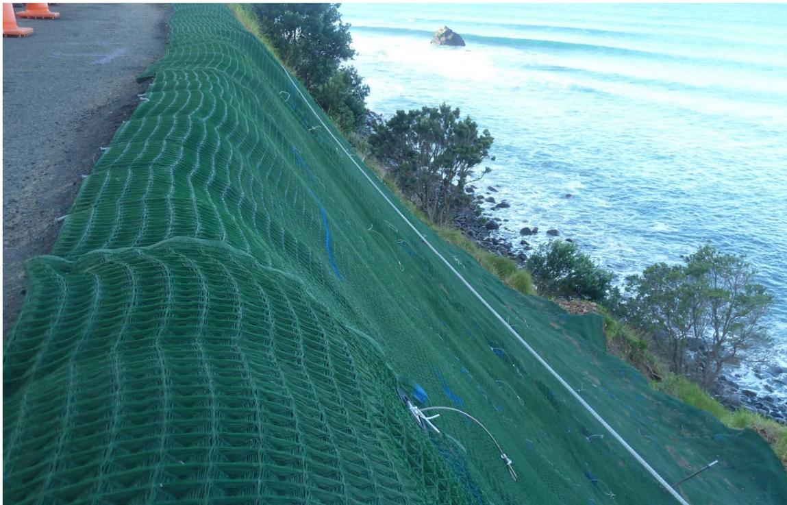
Figure 4.1B. Pyramat HPTRM Shoulder/Embankment Installation
