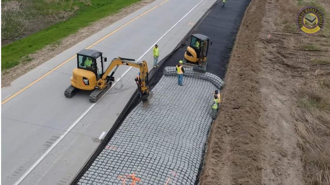
Figure 4.1A. Flexamat ACBM Installation Along Roadway Shoulder Prone to Overtopping
