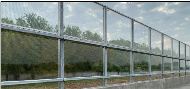
Test section of Acrylite Soundstop MASH TL-4 Noise Barrier System – image from Durisol testing information sheet
