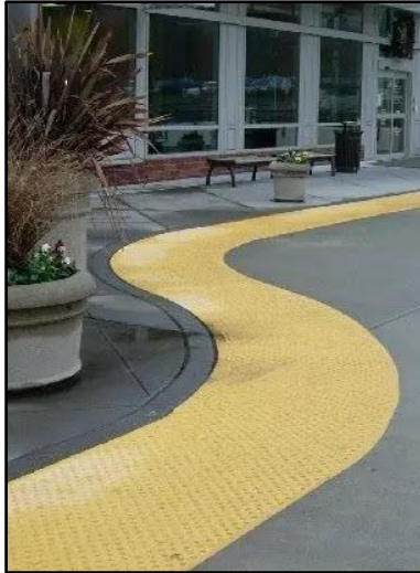
Example of Vanguard Nonskid Surface Applied Detectable Warnings installation with an irregular (curved) contour – image from Vanguard ADA Systems website
