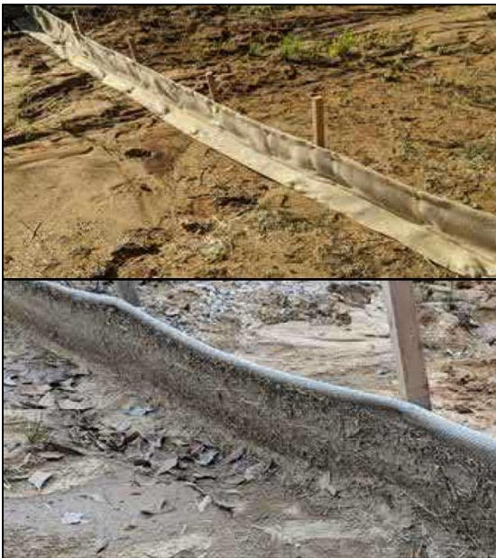
A new WattleFence™ installed on a jobsite (top), close-up of a WattleFence™ that retained eroded soils due to a large rain event (bottom) – images from Western Excelsior brochure
