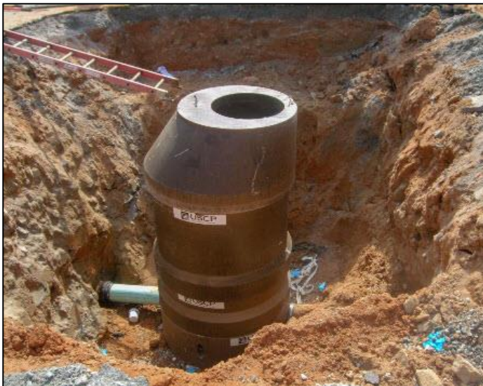
Installation of USCP Steel Reinforced Polymer Manhole – photograph from USCP website
