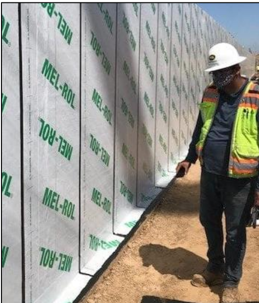
MEL-ROL being inspected on a recent installation – image from MEL-ROL website
