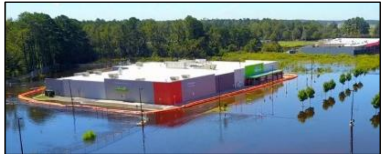
Tiger Dam™ protecting a Wal-Mart in North Carolina during a flood event – image from U.S. Flood Control Website
