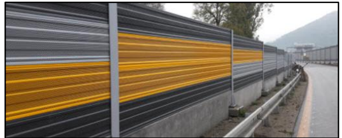
Durisol® Lightweight Aluminum Noise Barrier Panel – image from Durisol® website
