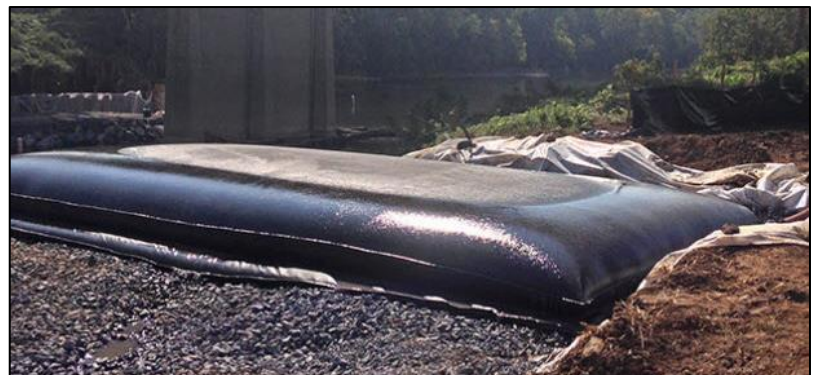
Example of a DirtBag®55 Dewatering Bag being used on a construction site – image from ACF Environmental website
