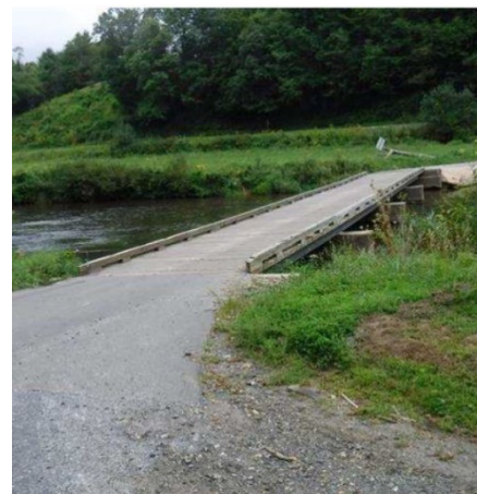
Figure 7: Timber curb that is typical on Project bridges
