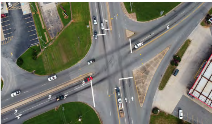
The Charlotte Rd/Railroad Ave intersection has dangerous crossing conditions for pedestrians
