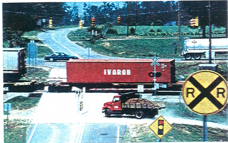
Signals, lights, gates and median barriers are some of the treatments used to improve safety at rail-highway crossings.
