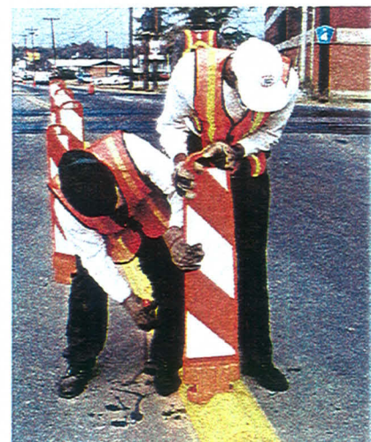
Installing median barriers
