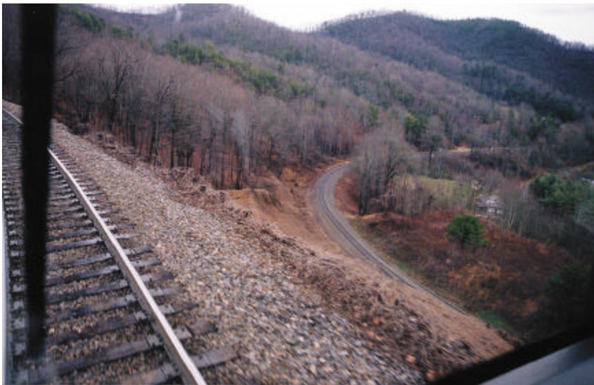
A partial view of 'the loops' between Old Fort and Asheville is seen from the locomotive. This curvy portion of railroad uses 12 miles to travel a straight-line distance of three miles.
