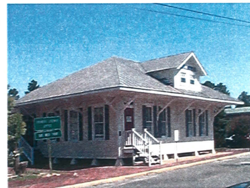
Mt. Olive — the former depot is now in use as a community center. The station was constructed about 1910.
