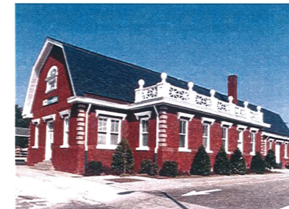
Fayetteville — four daily trains currently stop at the 1911 station. Construction of a new canopy and boarding platform is slated for 2005.
