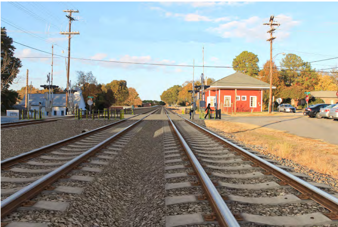
Pedestrian crossing safety, including gates and fencing, would be necessary and required for the new three-track corridor configuration.
