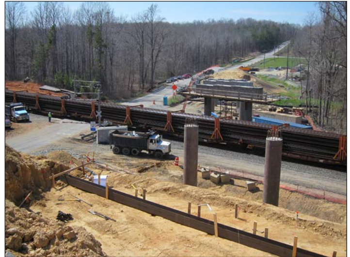
C-4901 Bowers to Lake - Upper Lake Road overpass
