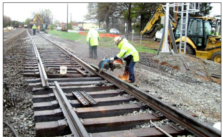
Detour cut in at Klumac Road
