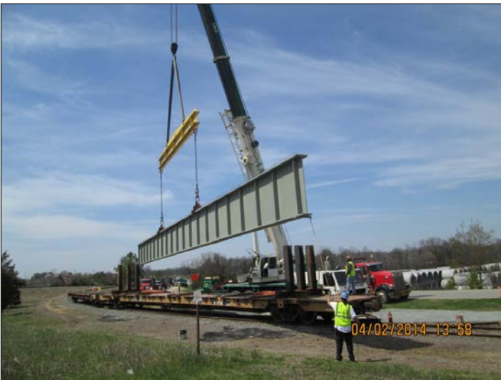
P-5208 Haydock to Junker - Bridge girder delivery
