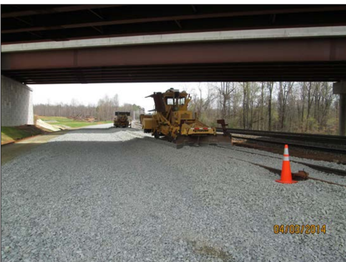
I-2304 Duke Curve Realignment - Complete Roadbed
