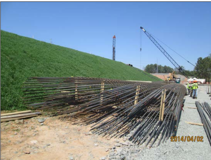
U-4716 Hopson Rd./Nelson-Clegg Structural materials
