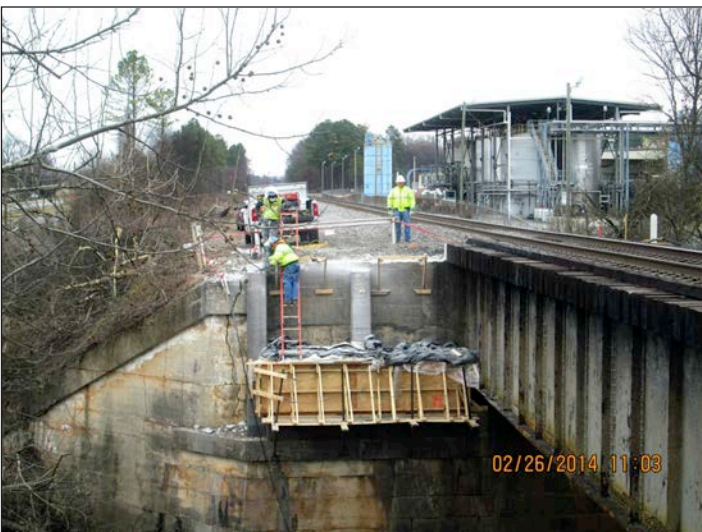
P-5208 Haydock to Junker - Bridge prep
