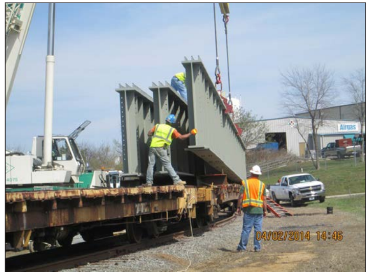
P-5208 Haydock to Junker - Bridge girder delivery
