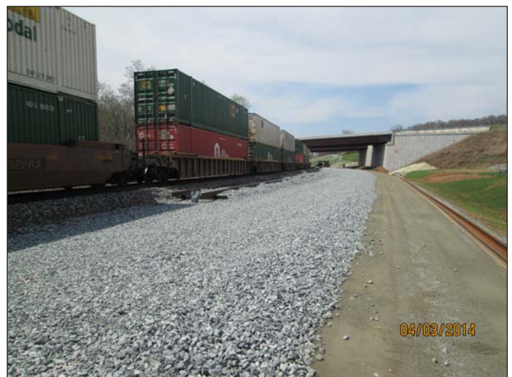
I-2304 Duke Curve Realignment - Ballast Pad
