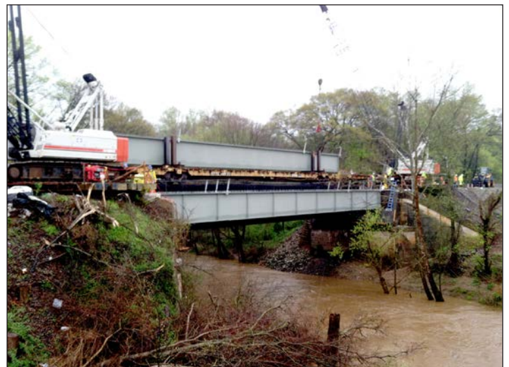
P-5208 Haydock to Junker - Bridge Girder Delivery
