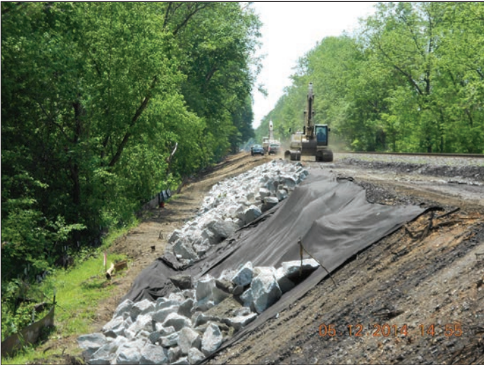
C-4901 Bowers to Lake - embankment stabilization
