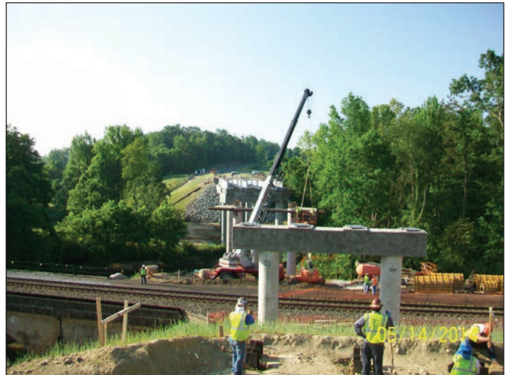
C-4901 Bowers to Lake - Turner Road overpass
