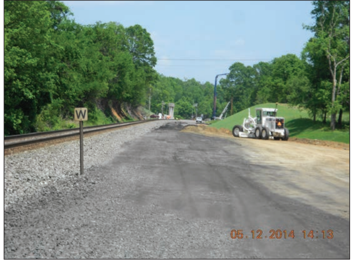
C-4901 Bowers to Lake - grading
