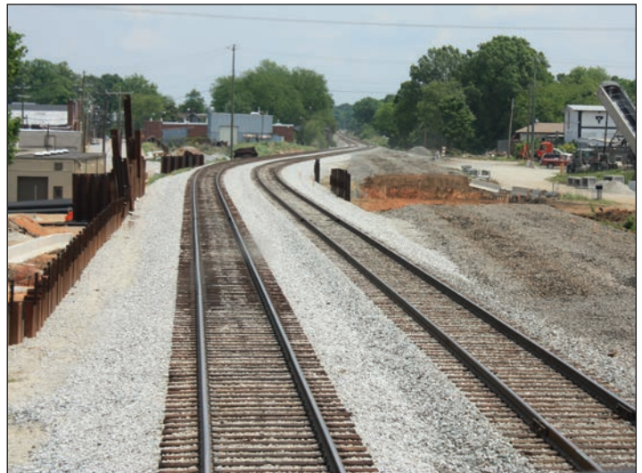
U-3459 Klumac Road - Detour tracks in place
