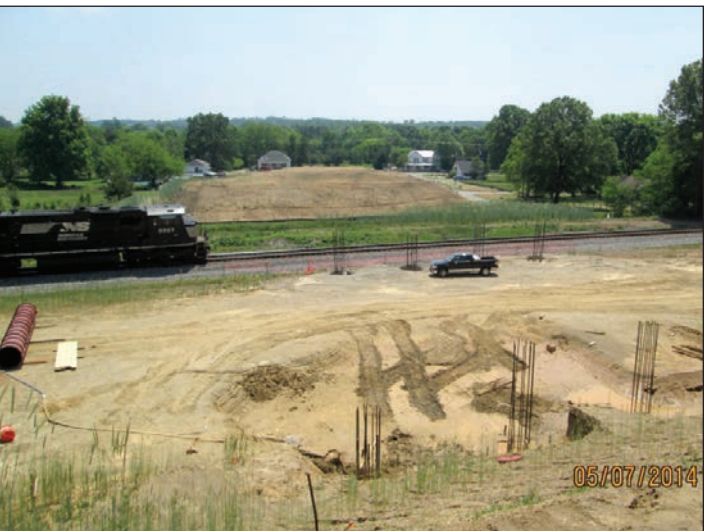
P-5208 Haydock to Junker - Roberta Road overpass
