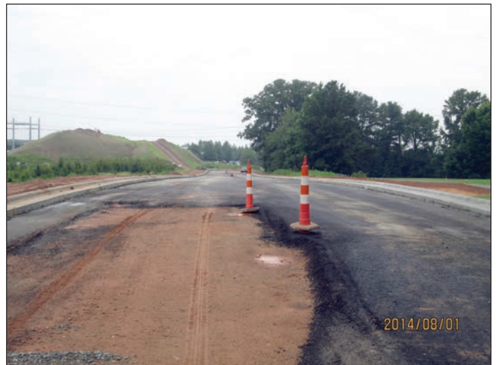
U-4716 Nelson to Clegg, Church Street Extension
