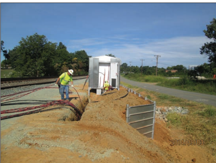
P-5205 Graham to Haw River, signal installation
