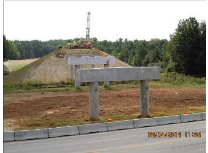
P-5206 Peeler Road Bridge Construction
