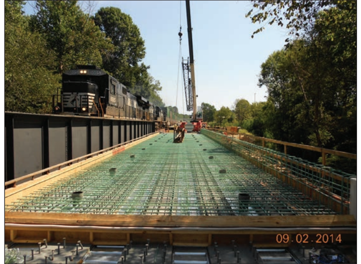
C-4901 Bowers to Lake - Bridge over Abbotts Creek
