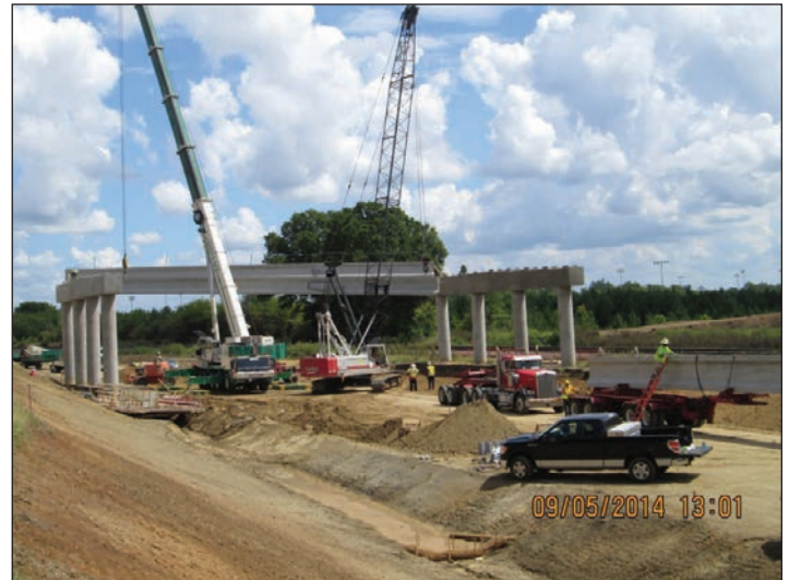
P-5208 Haydock to Junker - Roberta Road Grade Separation
