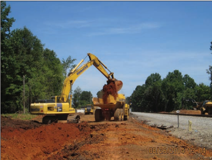
P-5206 Reid to N. Kannapolis - Ditching
