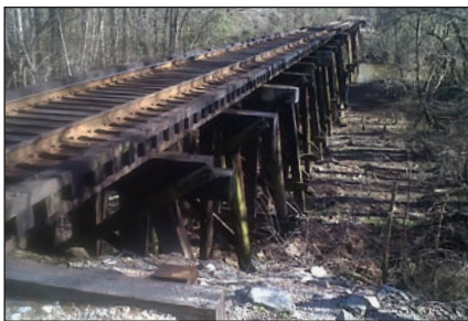
Meherrin River Bridge
