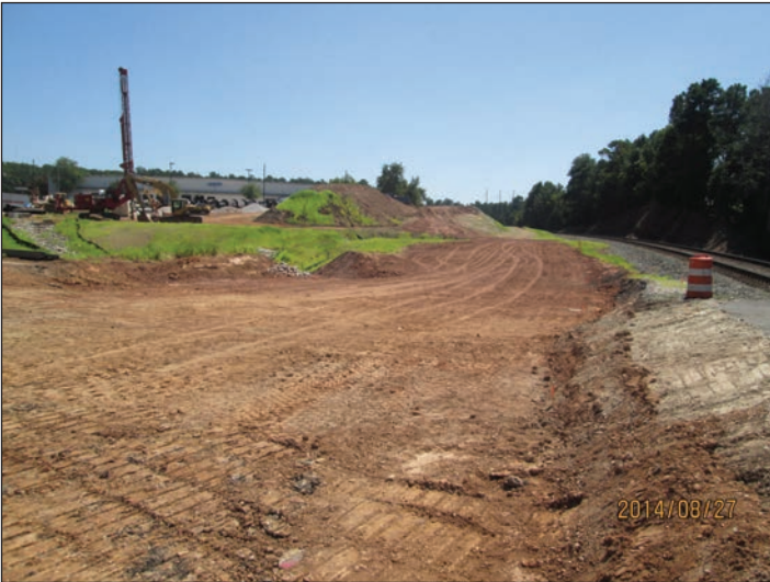
P-5201 Morrisville Parkway grading
