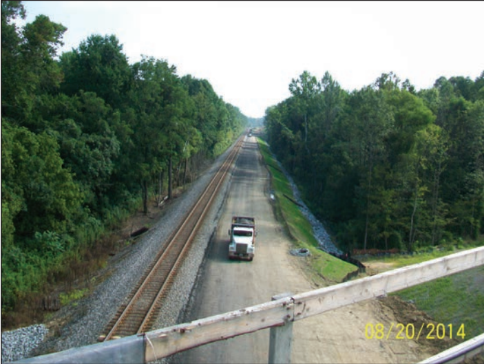
C-4901 Bowers to Lake - View from Upper Lake Bridge
