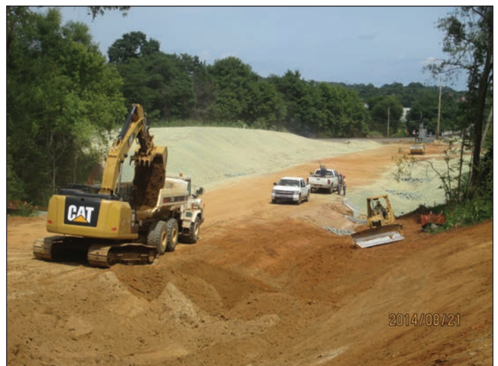
P-5205 Graham to Haw River Grading
