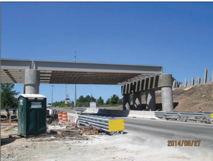
U-4716 Hopson Road bridge construction
