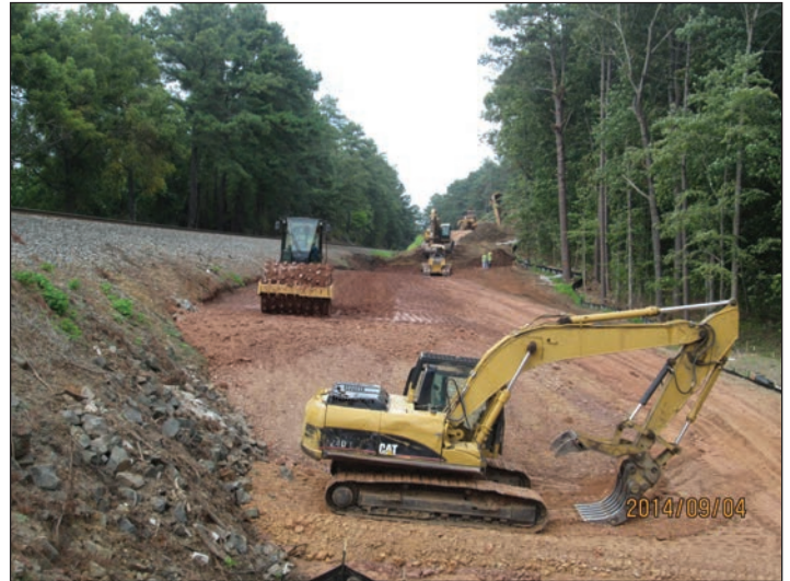
P-5201 Morrisville Parkway, west approach to bridge
