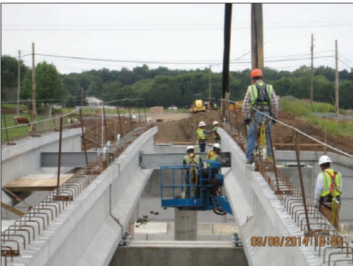
P-5208 Haydock to Junker - Pharr Mill Road Bridge
