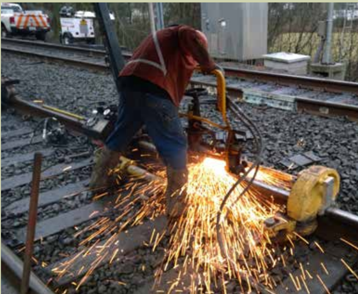
Rail repair in Washington State.
