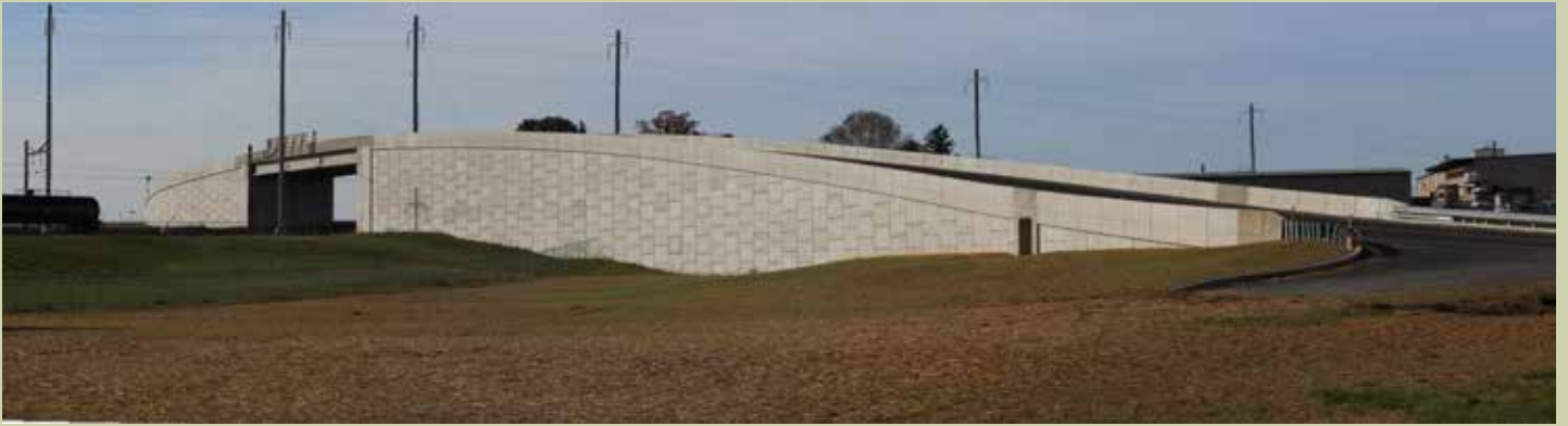
Lancaster County, PA, Eby Chiques Bridge; single span concrete I-beam bridge over Amtrak & Newcomer Road
