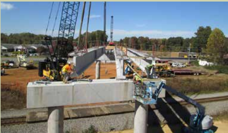
Bridge girders are being set for the Peeler Road Bridge, one of 12 Piedmont Improvement Program grade separation projects in North Carolina.
