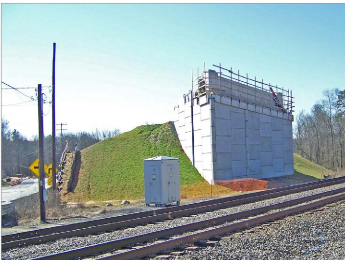
P-5204 McLeansville Road Bridge Construction
