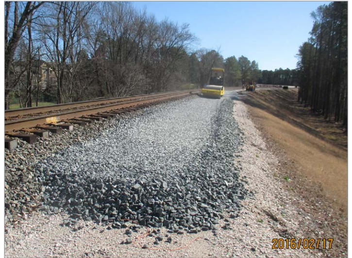
P-5201 Morrisville Parkway, track construction
