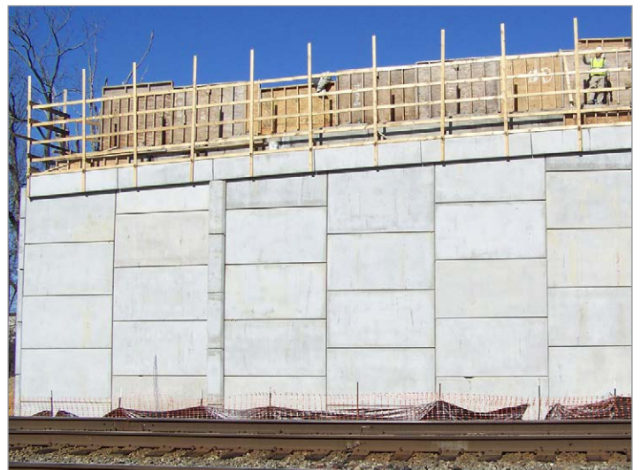
P-5204 McLeansville Road Bridge Construction
