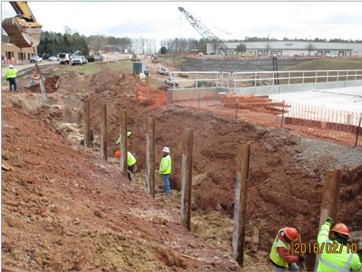
P-5201 Morrisville Parkway, bridge construction
