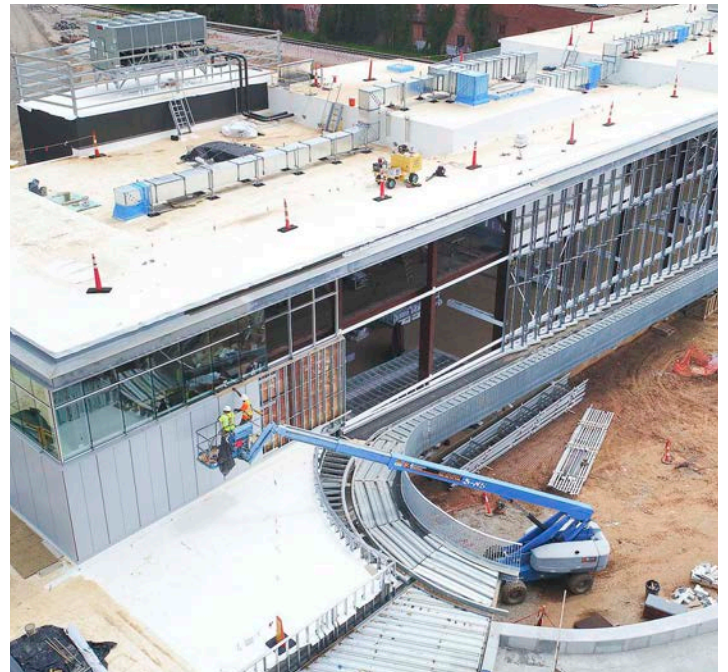
View of south elevation and installation of glazing
