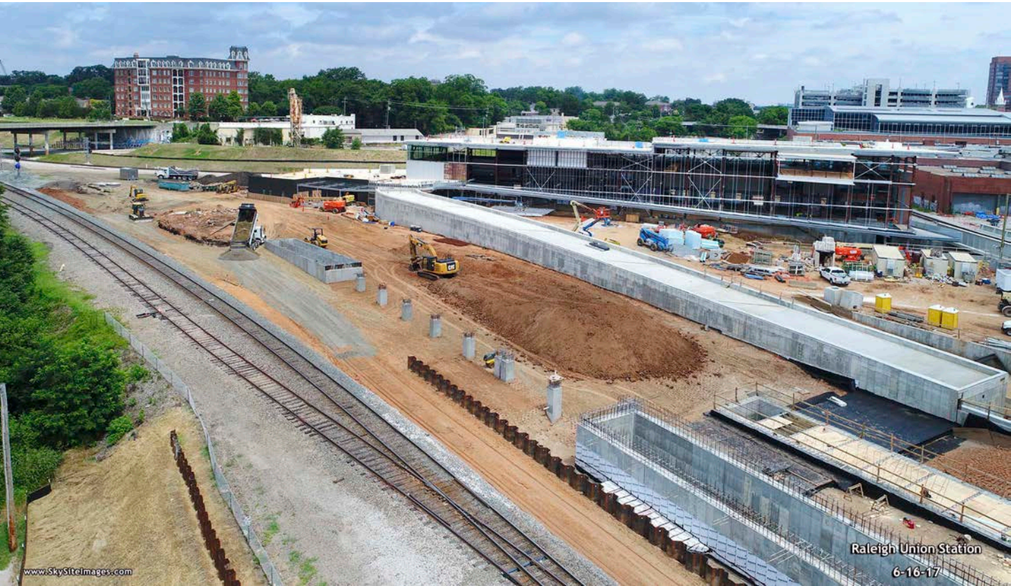
View of south elevation, with concrete passenger concourse and footings for platform and canopy in foreground
