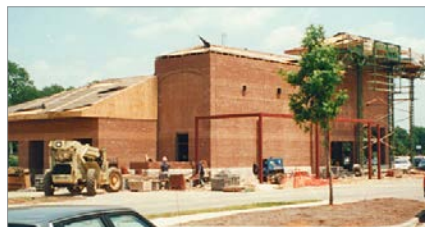
Station expansion underway, 2011
