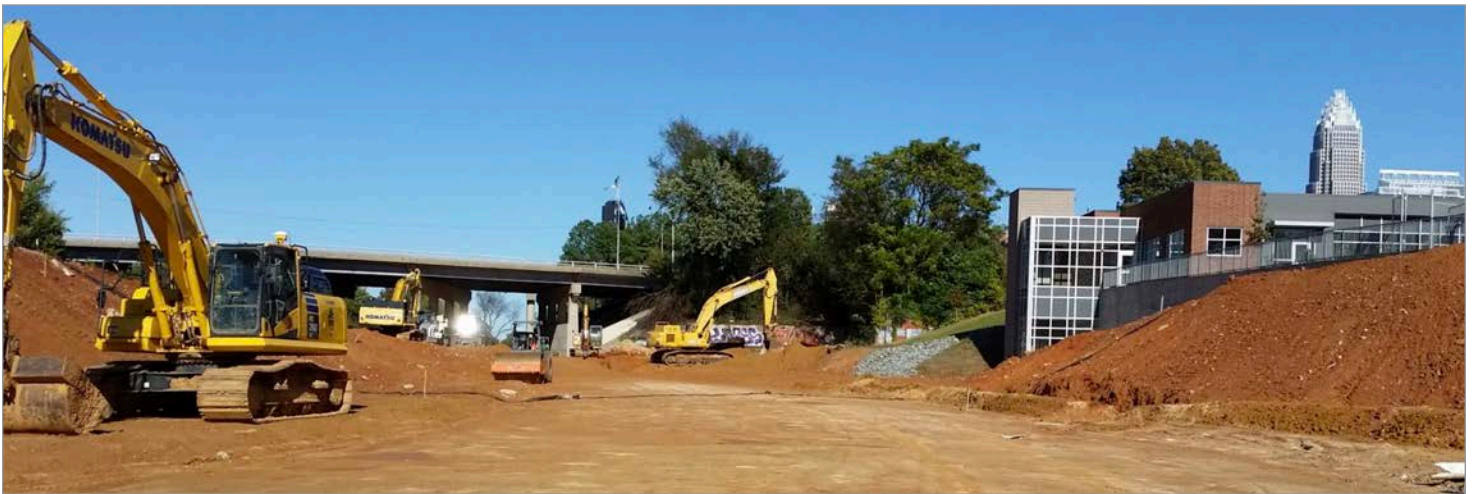
Grading for track
