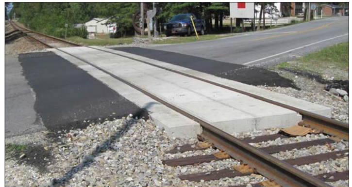
Brookside Camp Road after improvements
