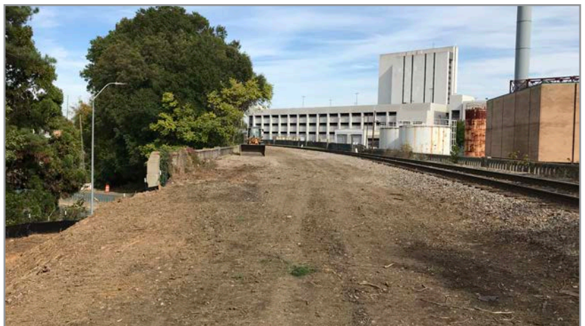
Lead track construction over Capital Boulevard bridge in Raleigh
