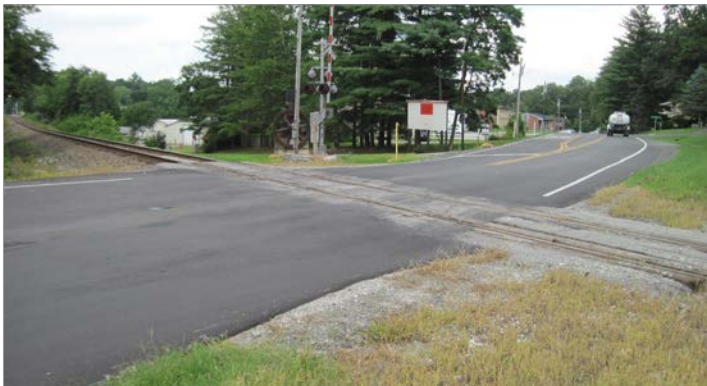
Brookside Camp Road before improvements
