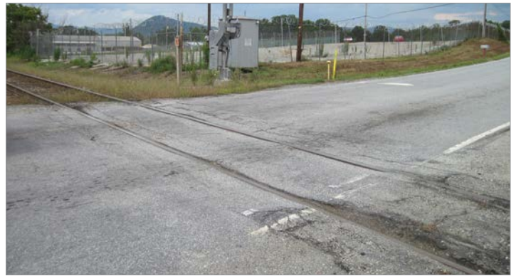
Brickyard Road before improvements
