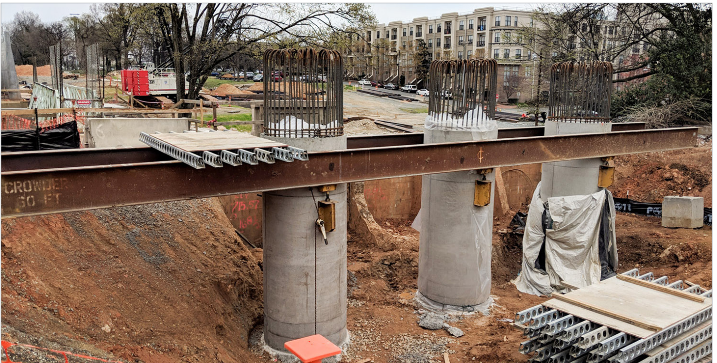
6th Street bridge pier column construction
