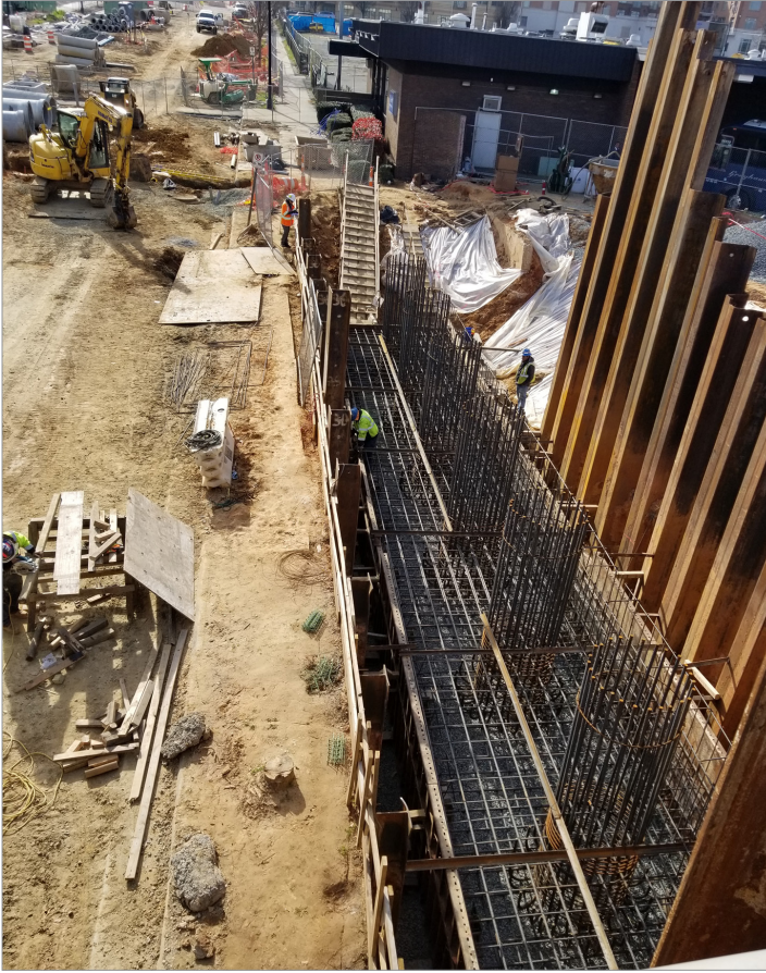
Trade Street bridge foundation pier construction
