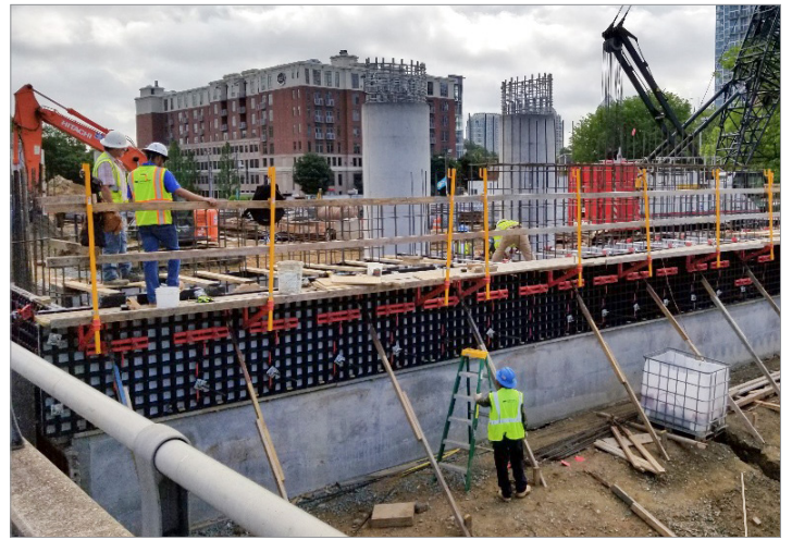
Trade Street end bent construction
