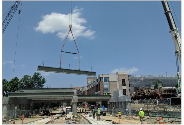
Girder installation at Trade Street, west view
