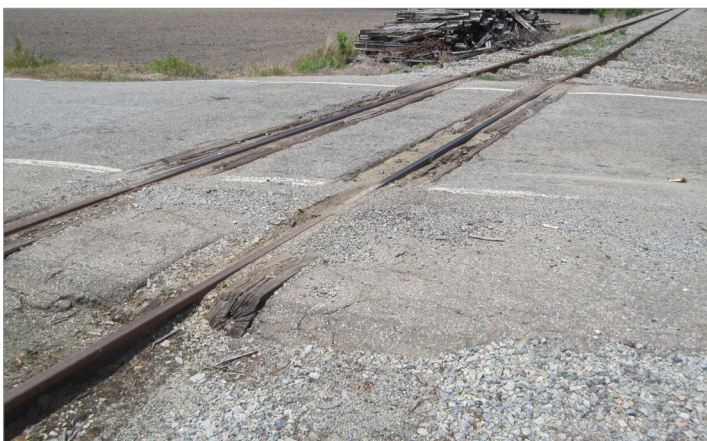
East Bear Swamp Road crossing before improvements
