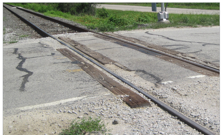
Donald Mercer Road crossing before improvements
