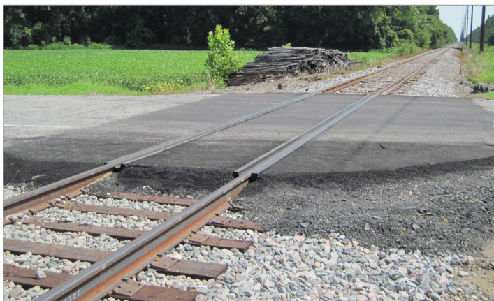
East Bear Swamp Road crossing after improvements
