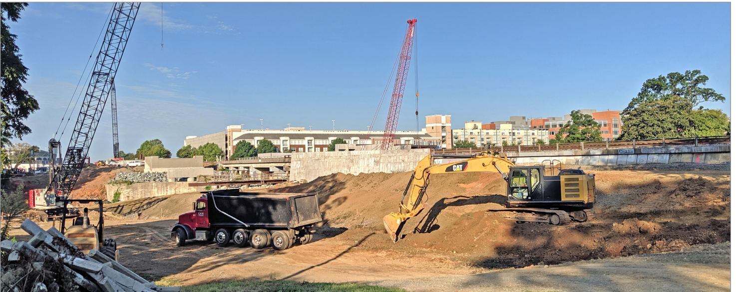
Grading between 6th and 7th Streets
