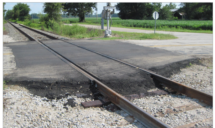
Donald Mercer Road crossing after improvements
