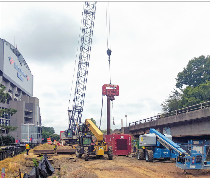
Bridge construction over pedestrian walkway
