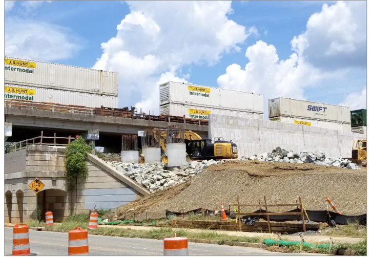
Bridge construction at 6th Street
