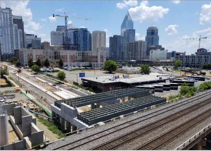
Bridge construction at Trade Street
