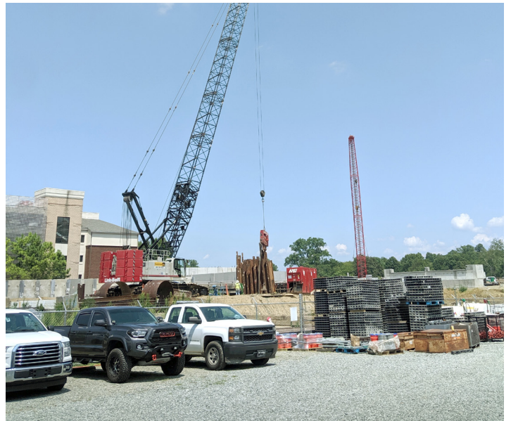
Bridge construction at 5th Street
