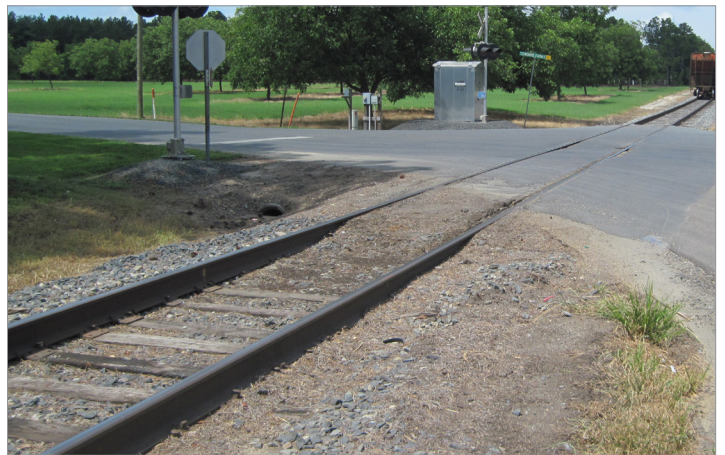
Morris Road crossing before improvements
