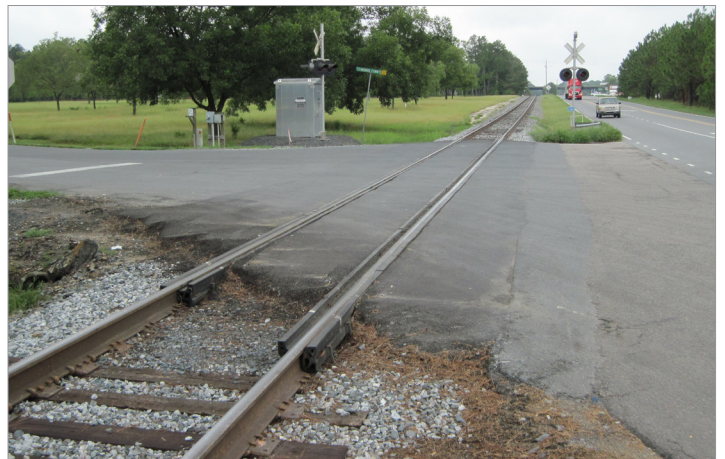
Morris Road crossing after improvements
