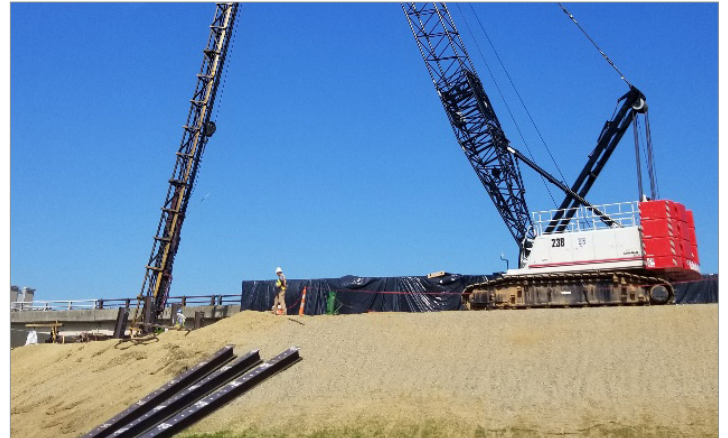
Bridge construction at 6th Street
