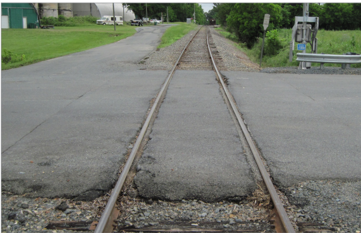
Anson Avenue crossing before improvements
