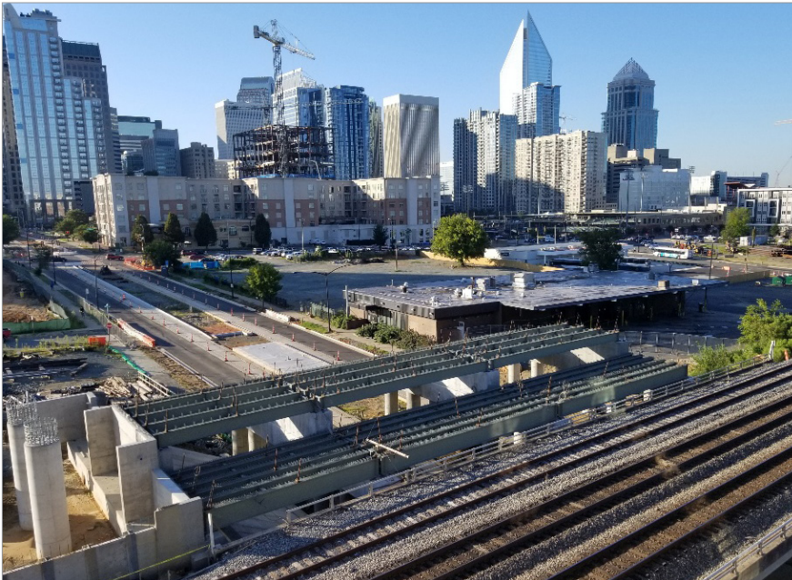
Bridge construction at Trade Street
