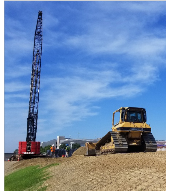
Grading between 6th and 7th Street
