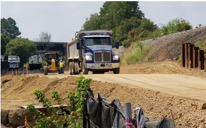
Subballast installation
