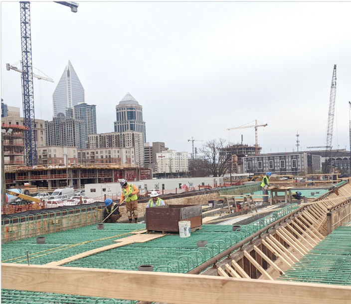
5th Street bridge deck construction
