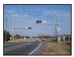
Example of gates, signs and flashing lights
