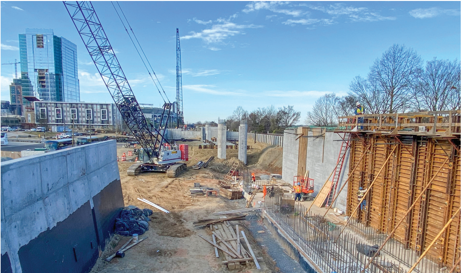
Construction of concourse foundation
