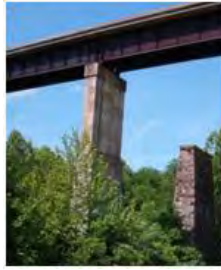
TAR RIVER BRIDGE
