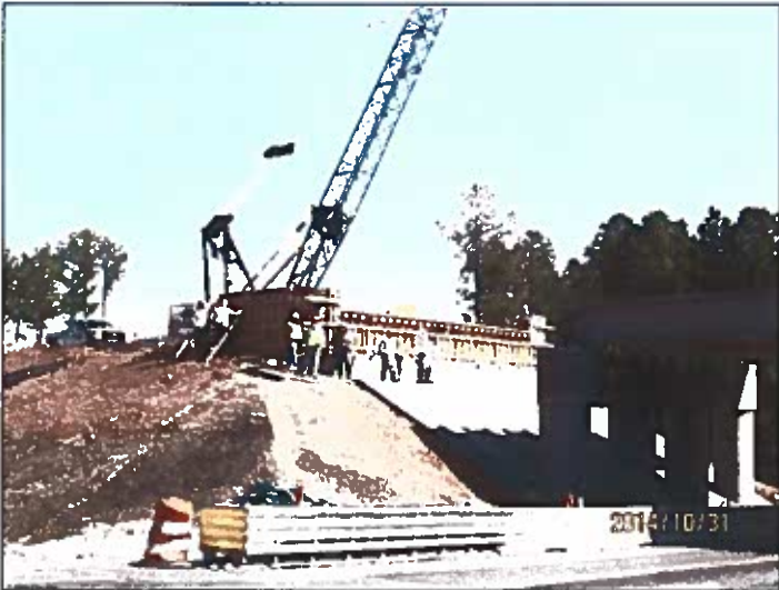
U-4716 Hopson Road bridge construction
