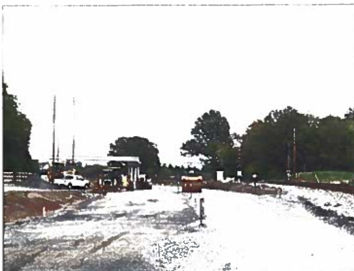
P-5208 Haydock to Junker - Roberta Road Bridge
