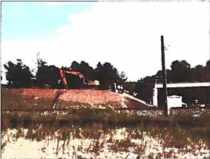
U-4716 Hopson Road bridge construction
