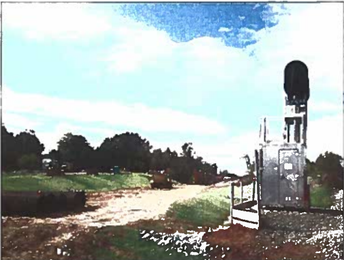
P-5205 Graham to Haw River Grading
