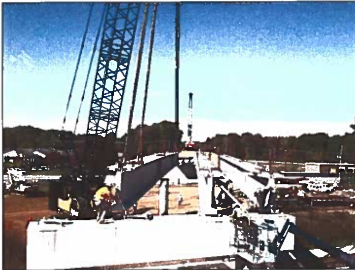
P-5206 Reid to N. Kannapolis - Peeler Road Bridge Construction
