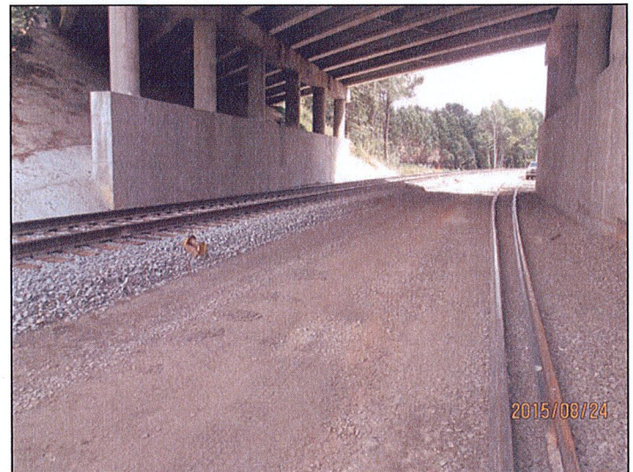
P-5500C Tryon Siding, roadbed ready for track construction
