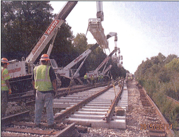
Congestion Mitigation Project, installation CP Armstrong turnouts
