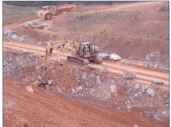
P-5205 Graham to Haw River Passing Siding, grading for new alignment
