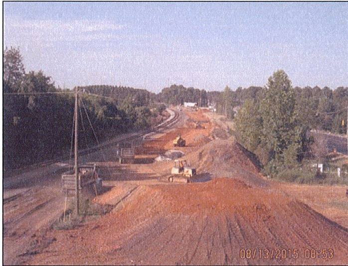
P-5206 Reid to North Kannapolis, grading near Peeler Road
