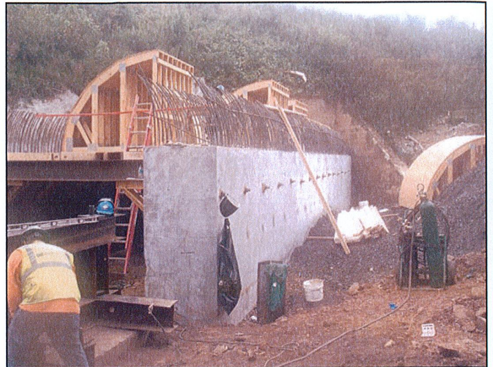
P-5208 Haydock to Junker, Arch culvert construction
