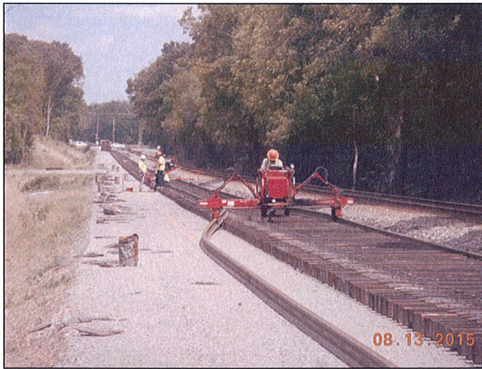
P-5208A Haydock to Junker, track construction
