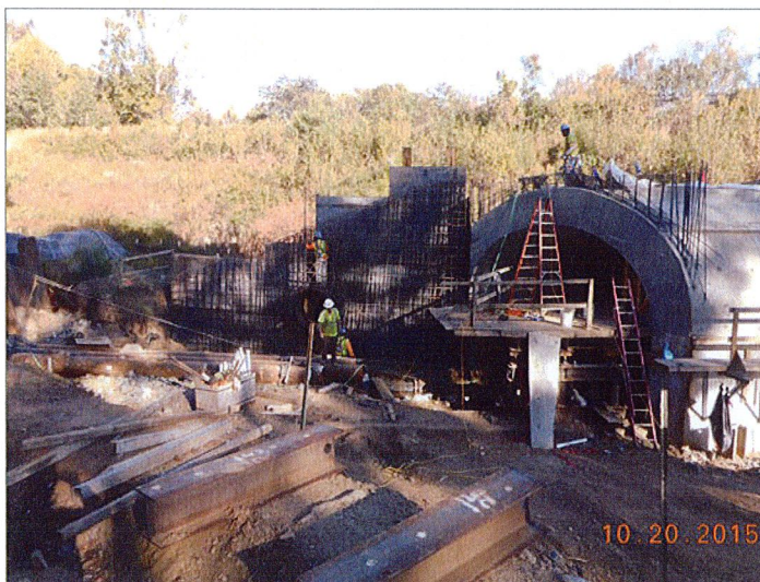
P-5208 Haydock to Junker, arch culvert construction
